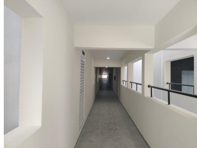
COMMON AREA ALL FLOOR CLEANING COMPLETED
