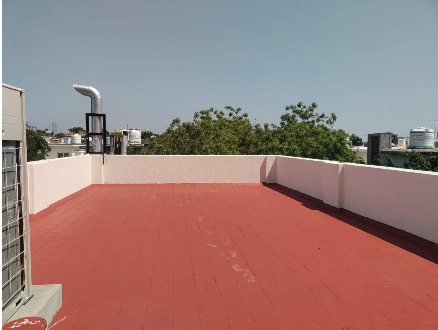
AMENITY BLOCK TERRACOTTA PAINTING COMPLETED
