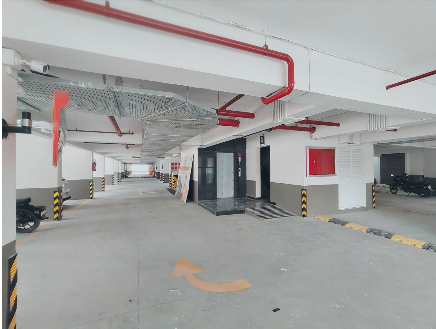
STILT FLOOR - COMPLETED
