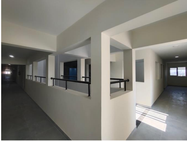
COMMON AREA ALL FLOOR CLEANING COMPLETED
