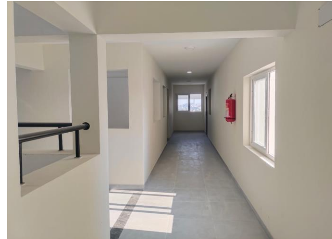
ALL COMMON AREA WORKS COMPLETED
