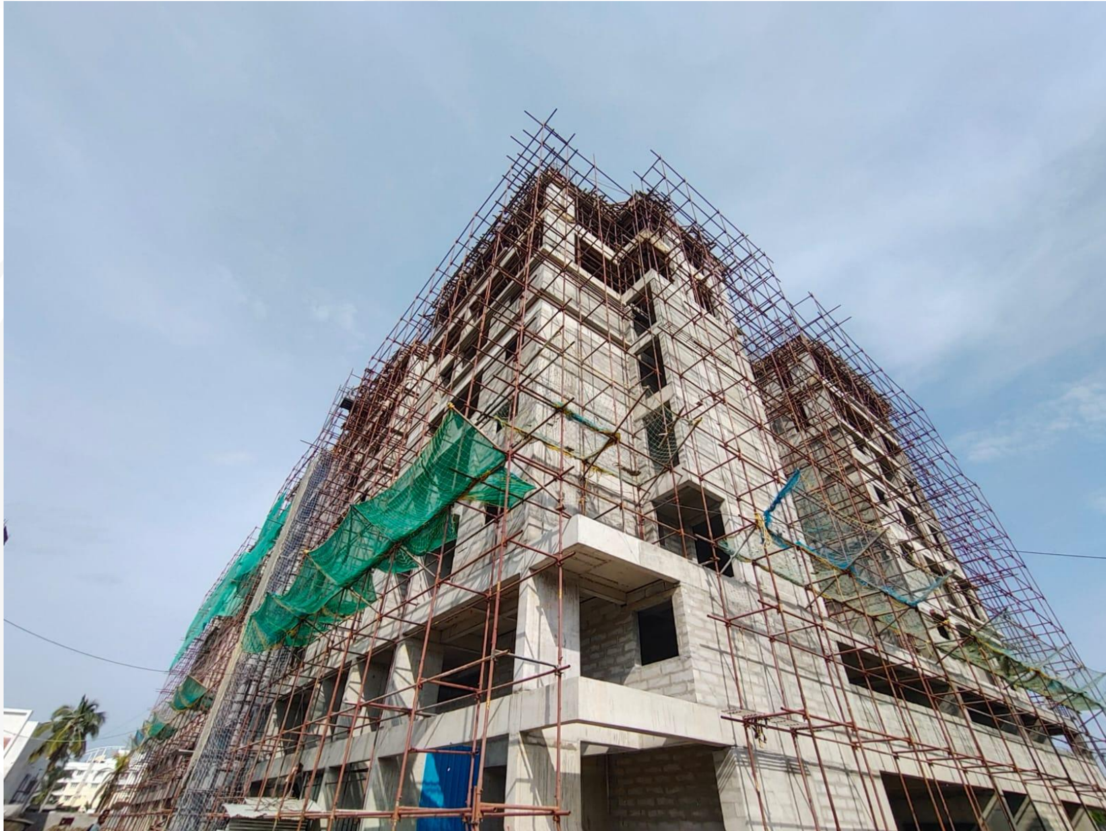
Main Building – North West Side View.
