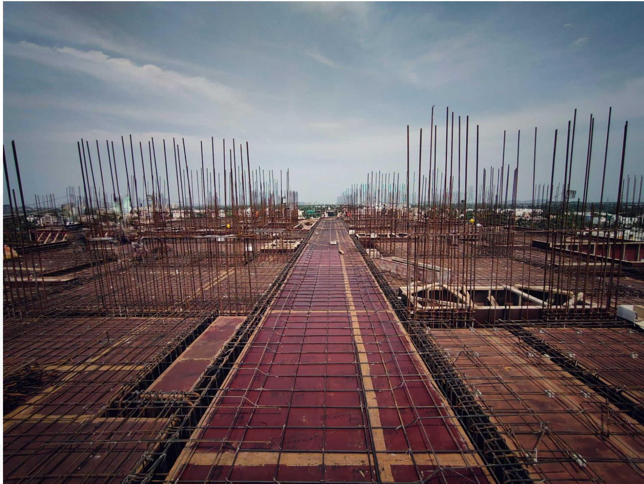
Main Building – Seventh Floor Slab Reinforcement Work In Progress
