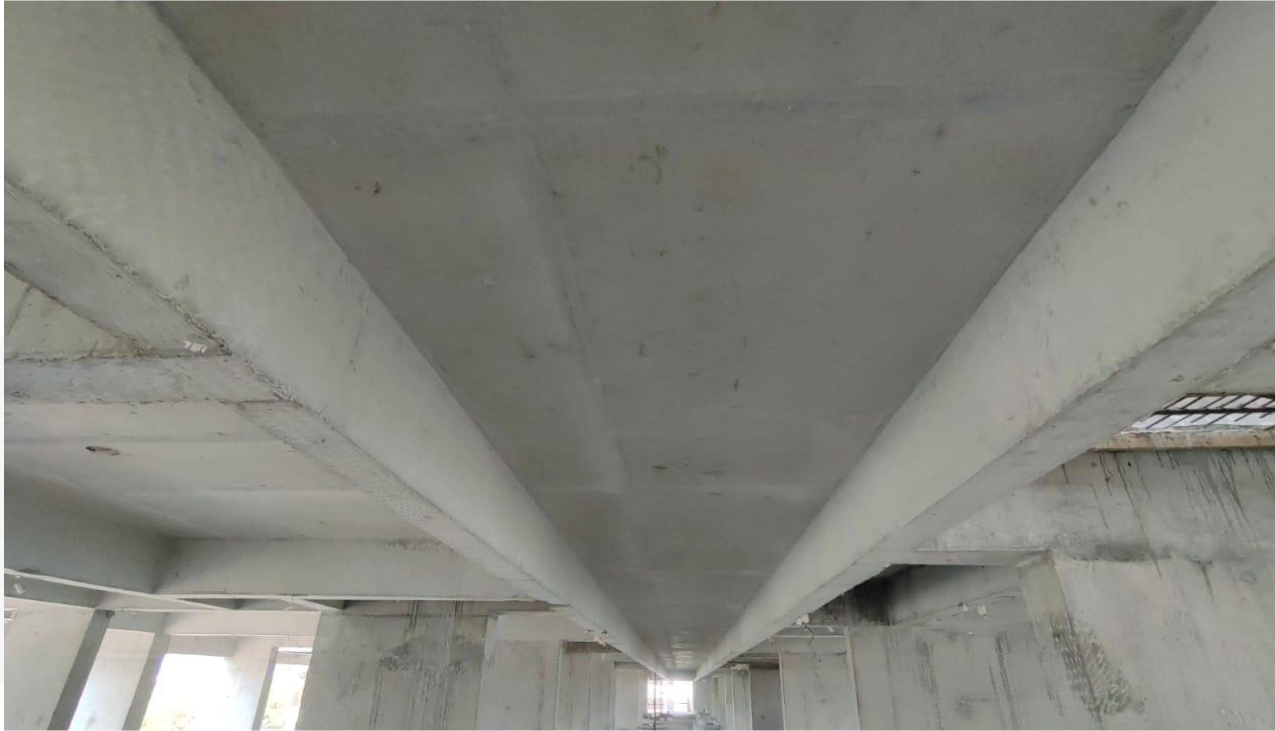
Fifth Floor– Hacking work & surface grinding work in progress.
