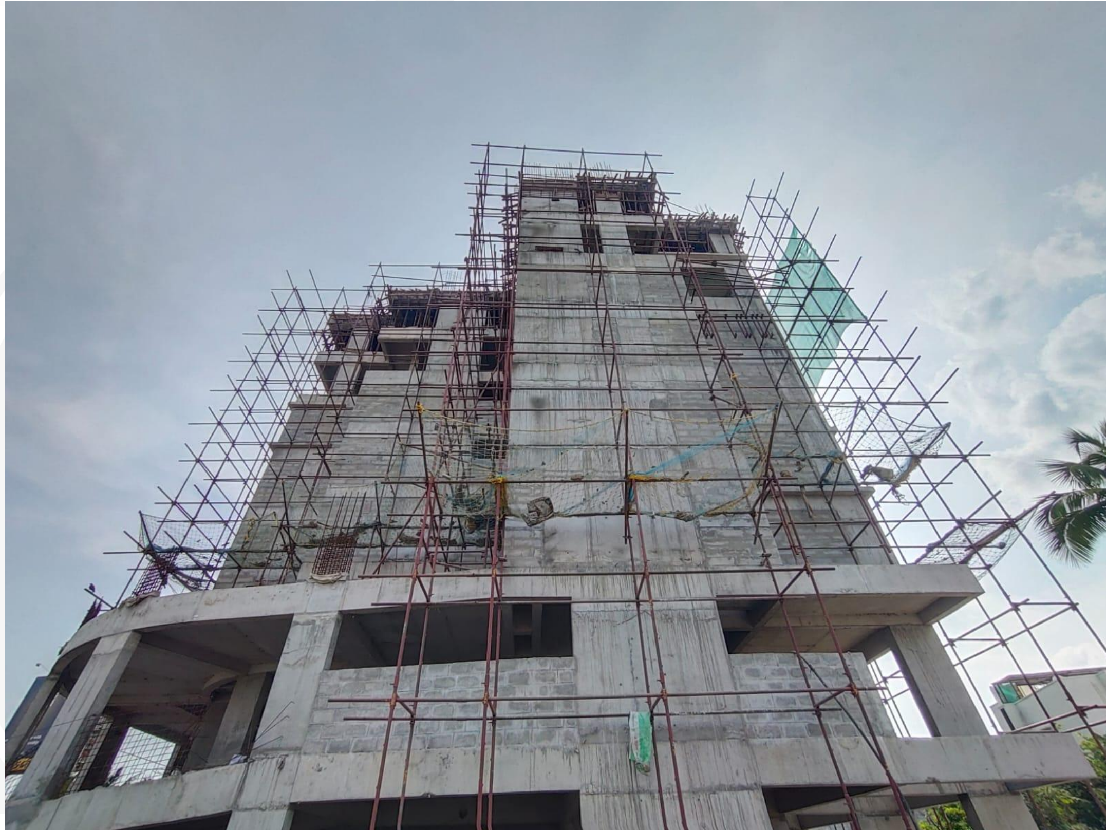
Main building – East side view.
