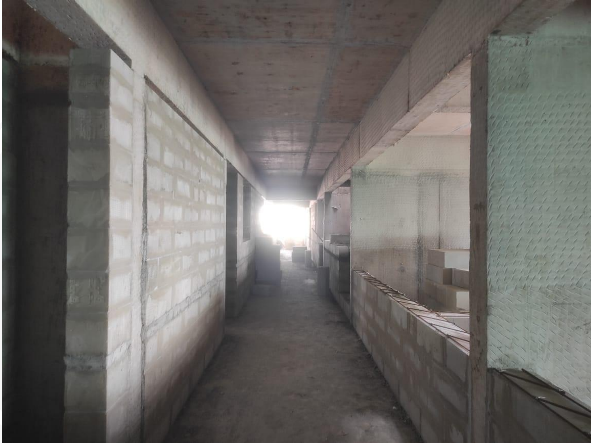
Fourth Floor – Block work In Progress
