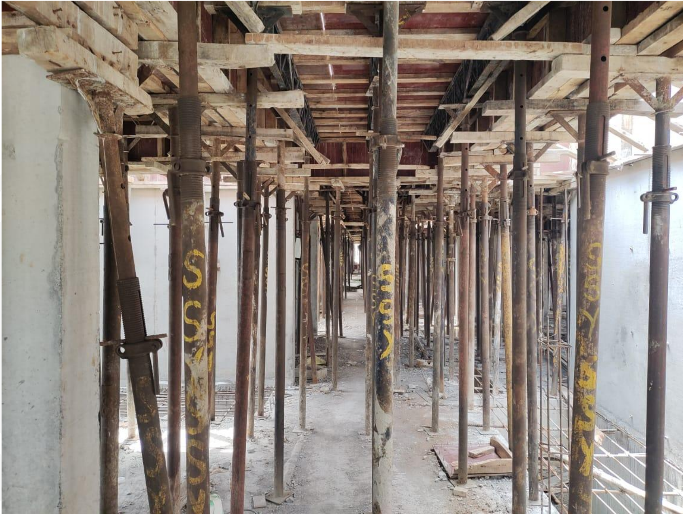
Main Building – Seventh Floor Shuttering Work In Progress
