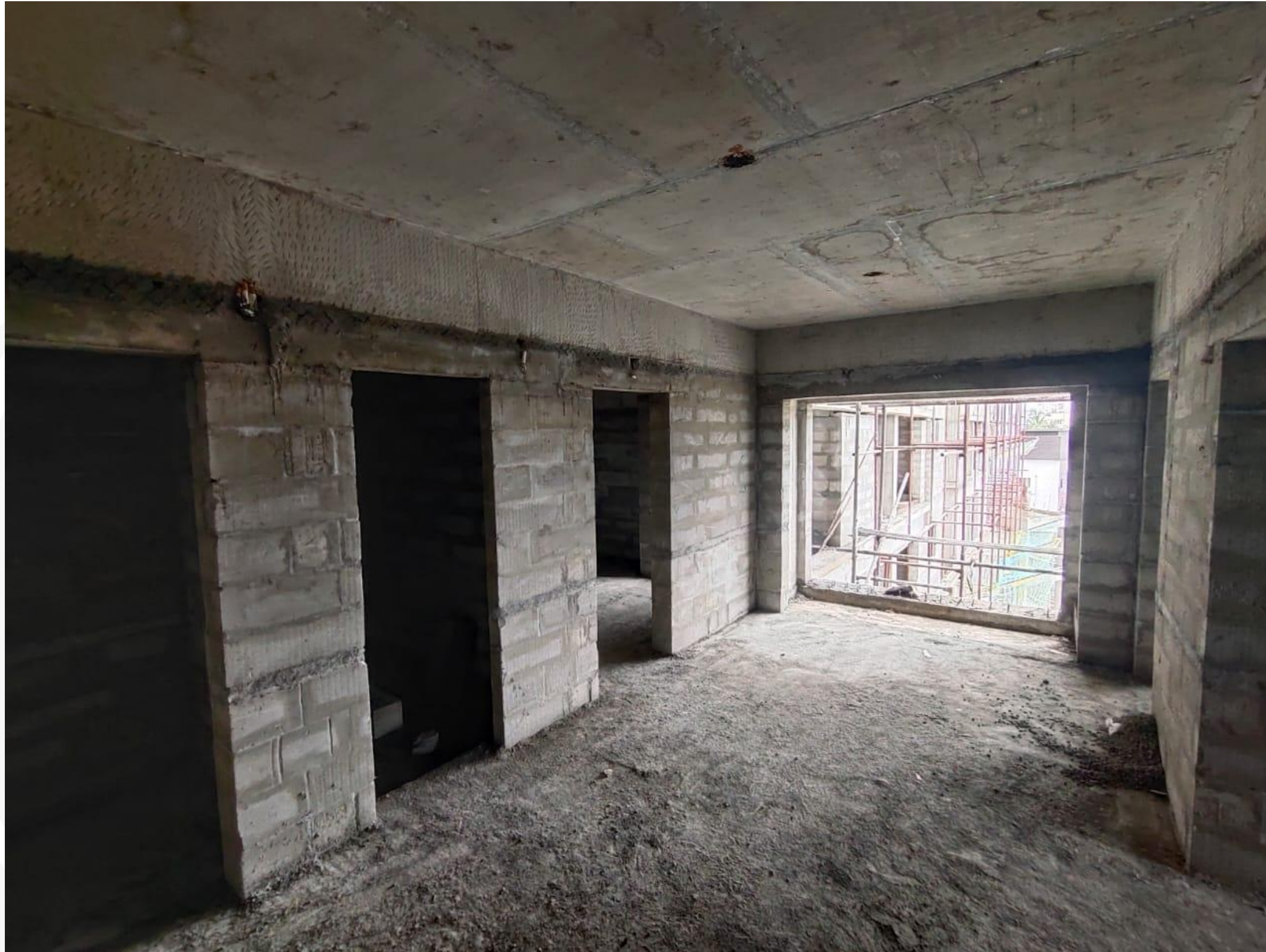
Second Floor – Block work Is Completed
