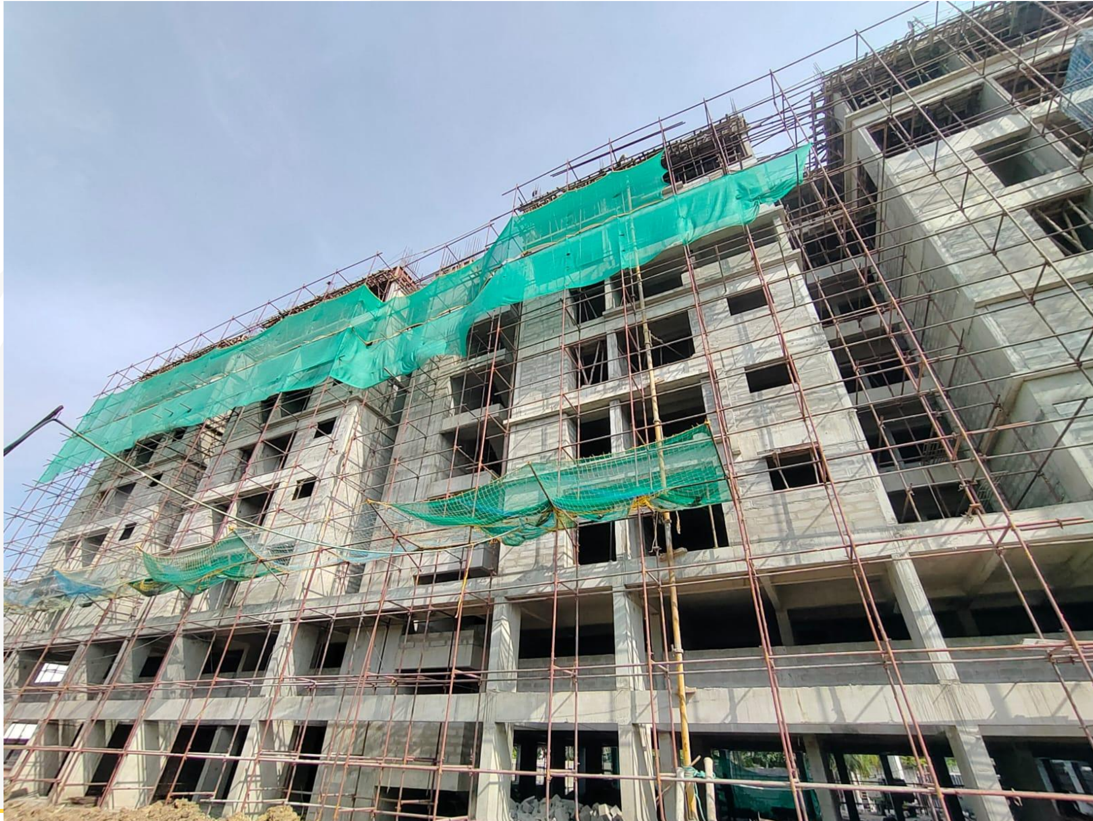
Main Building– North Side View
