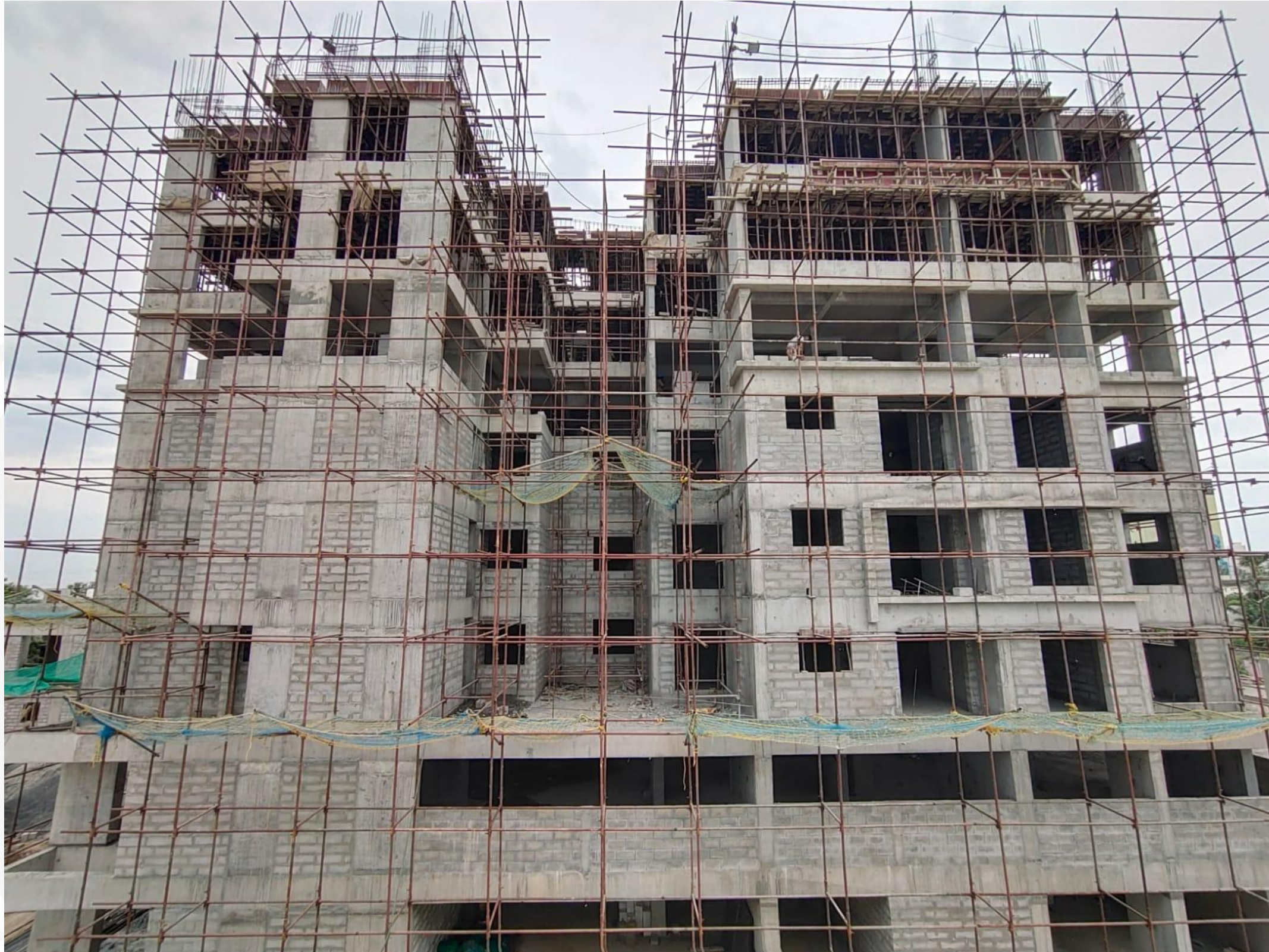
Main Building – Seventh Floor Slab Shuttering & Reinforcement Work In Progress
