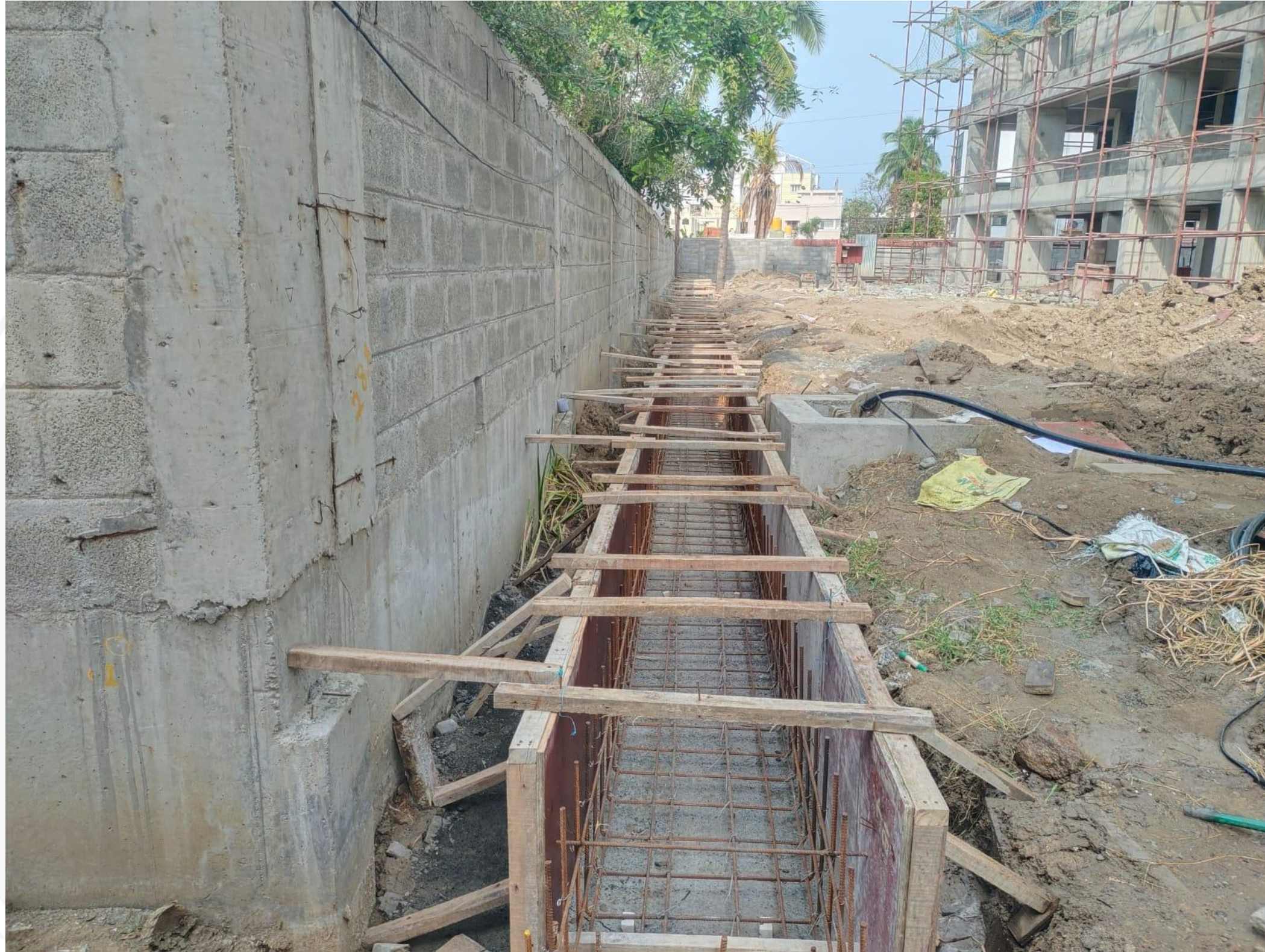
EXTERNAL TRENCH – Trench Raft & Wall Reinforcement Work In Progress.
