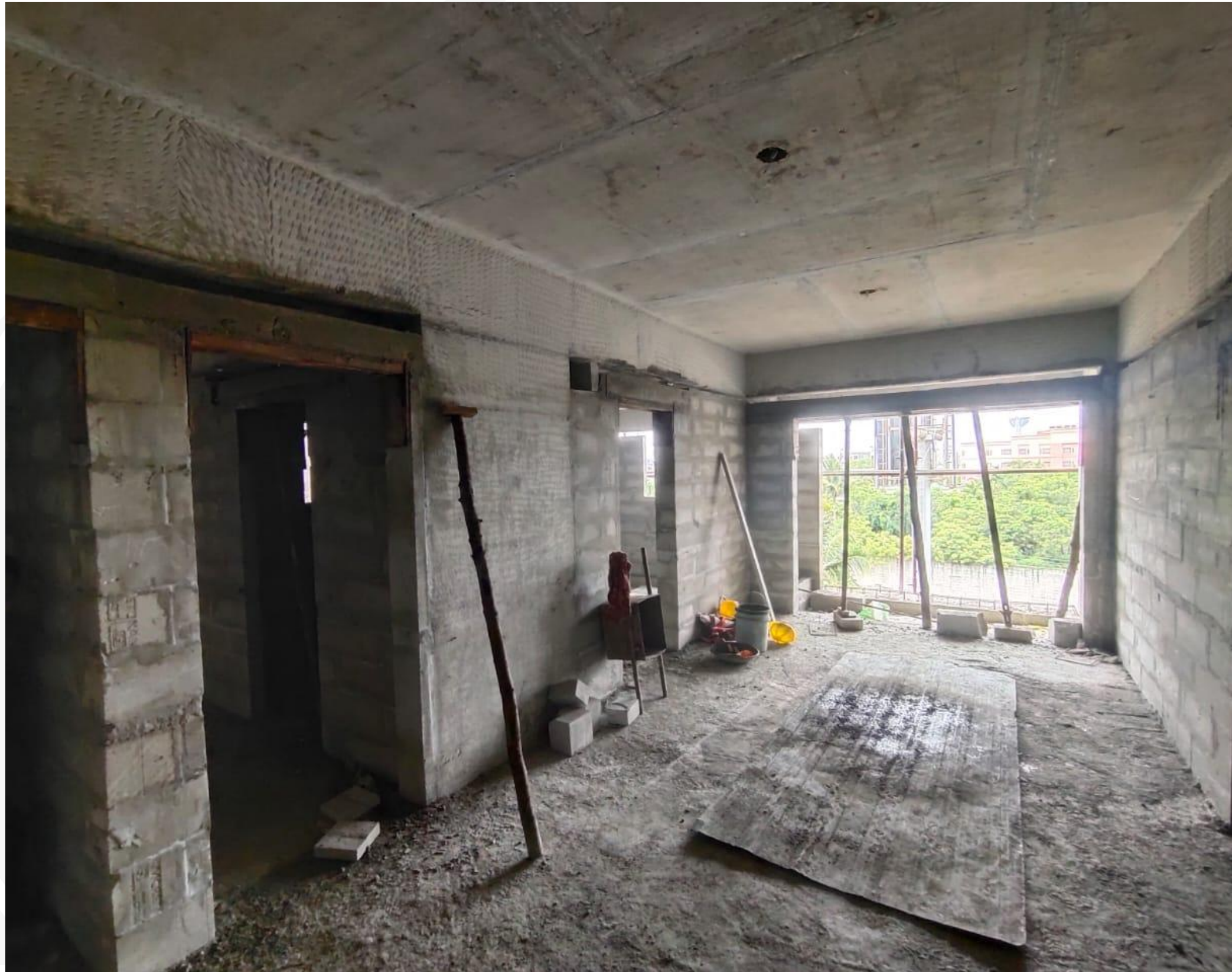
Third Floor – Block work In Progress
