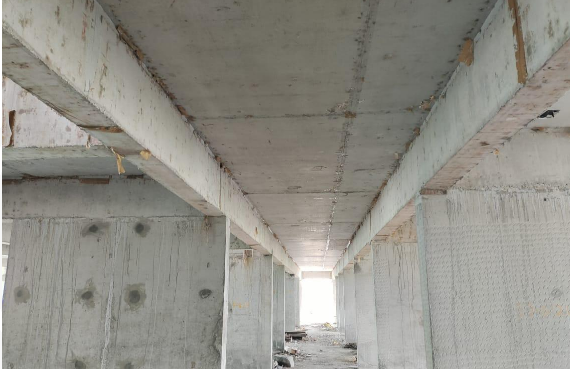
Main Building – Sixth Floor Slab De-Shuttering Work Completed
