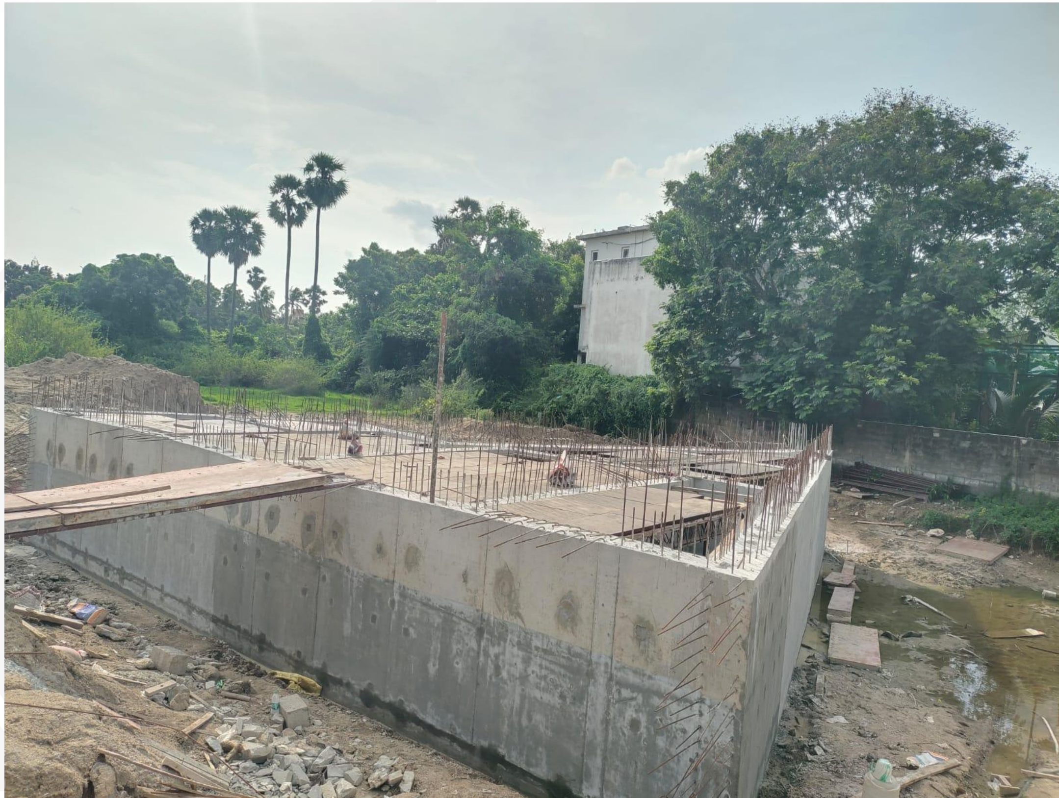
STP – Wall 2 nd lift waterproofing & Slab Shuttering Work In Progress
