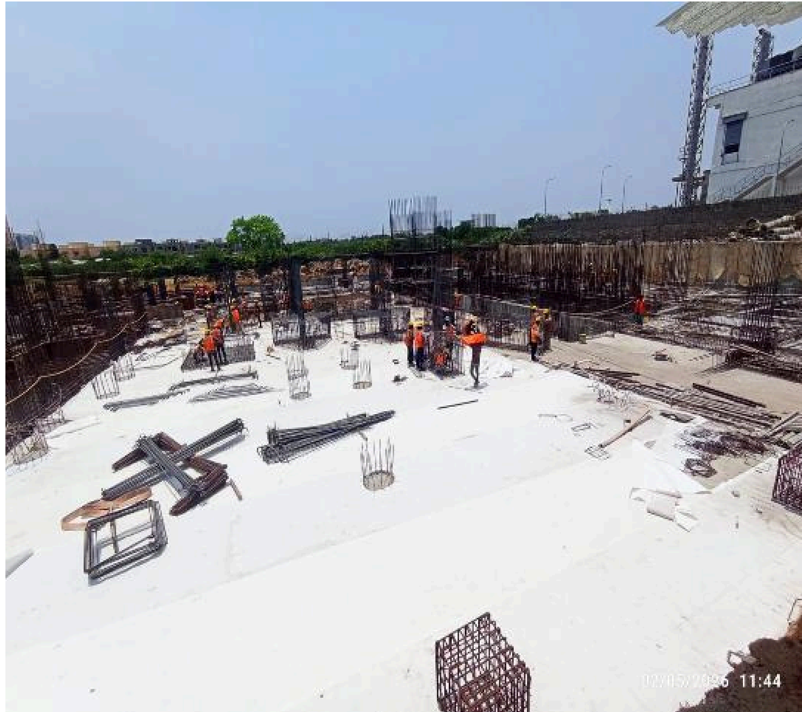
iHeart – Wing 2 Waterproofing and Pile Cap Reinforcement Work
