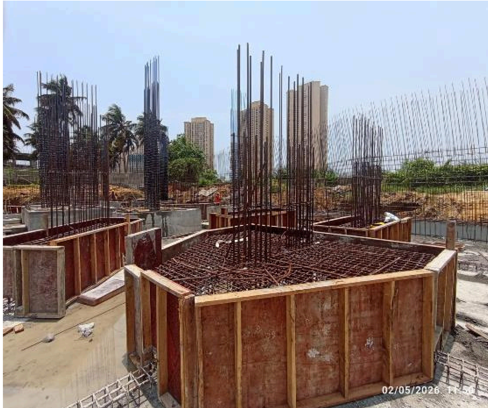
iHeart – Wing 2 Pile cap Reinforcement, Shuttering and Concreting Work
