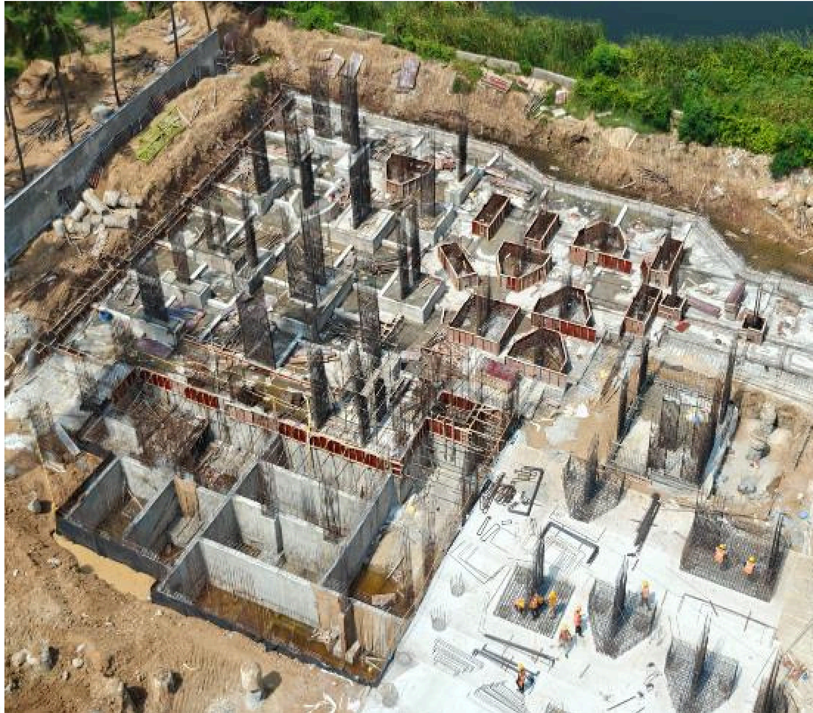
DRA iHeart – Wing 2 Pile Cap Shuttering and Water Proofing Work
