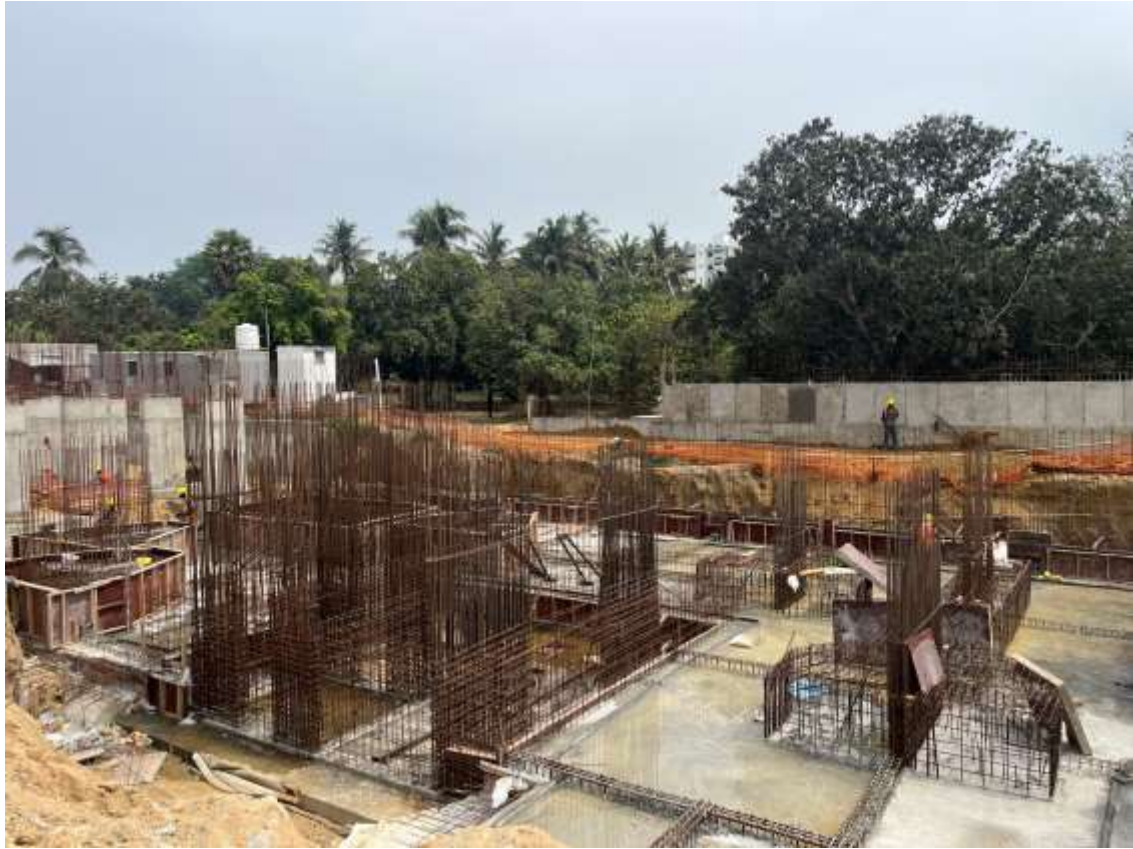
iHeart – PCC & Lift Pit Wall curing & Reinforcement Work
