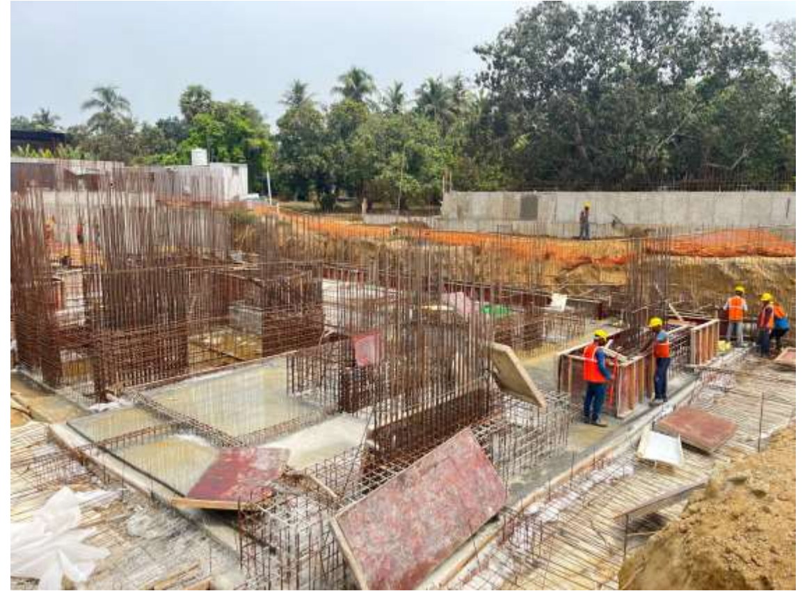
iHeart – PCC & Lift Pit Wall curing & Reinforcement Work
