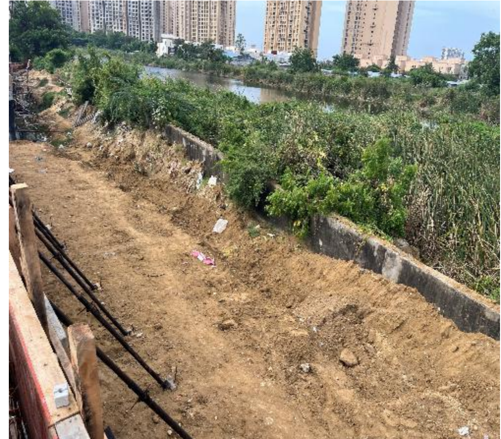
iHeart – Wing 1 Backfilling Work
