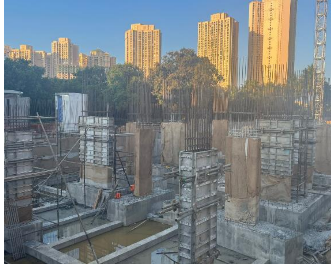
iHeart – Wing 2 Column Curing Work
