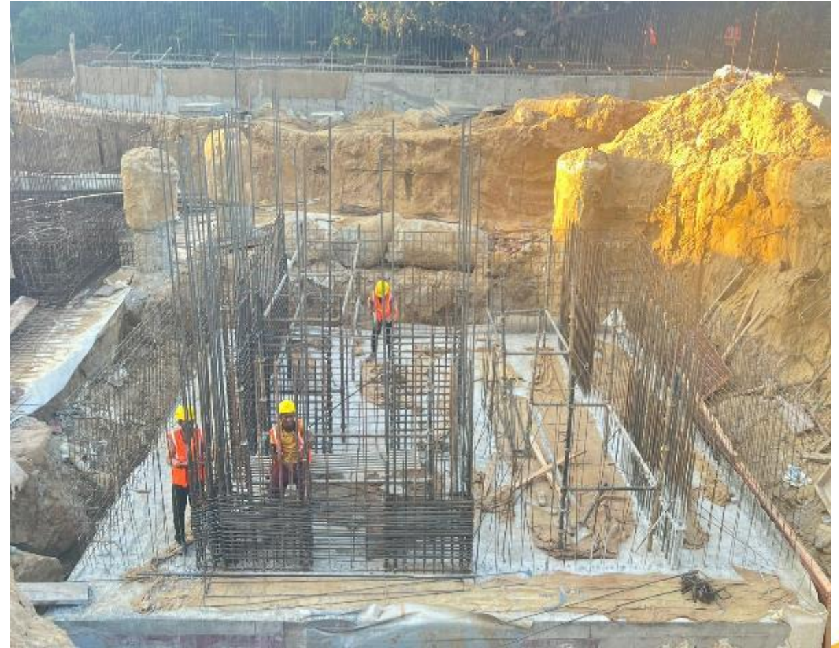
iHeart – Wing 1 PCC & Lift Pit Wall Reinforcement Work
