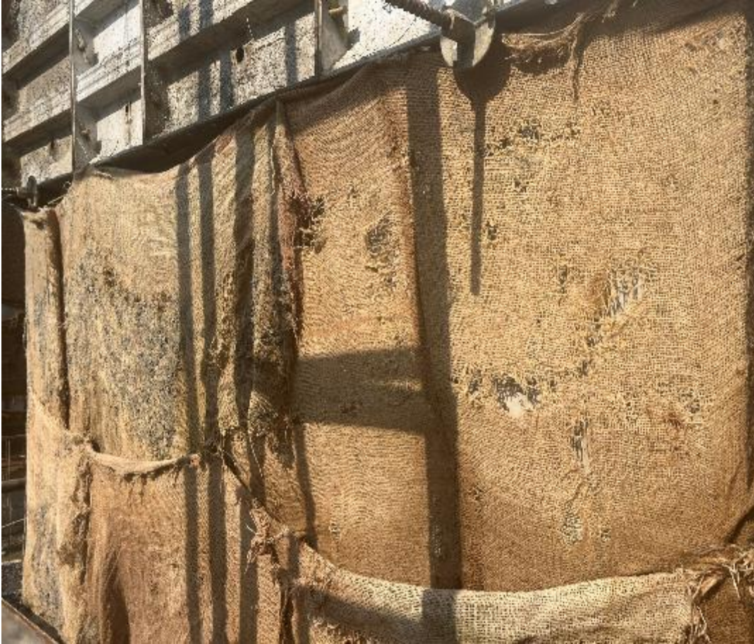
iHeart – Wing 2 Column Curing Work
