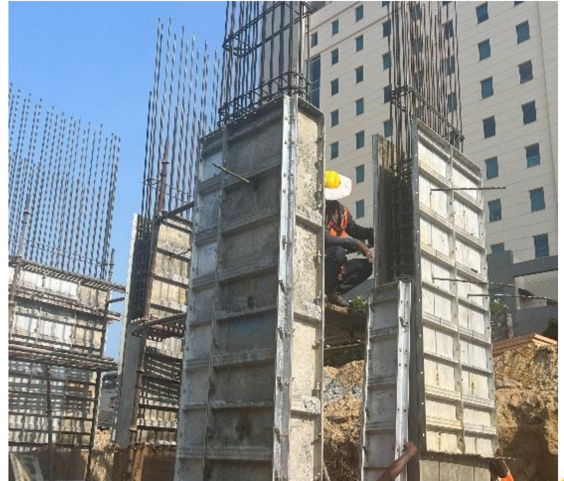
DRA iHeart – Wing 2 Column Shuttering Work
