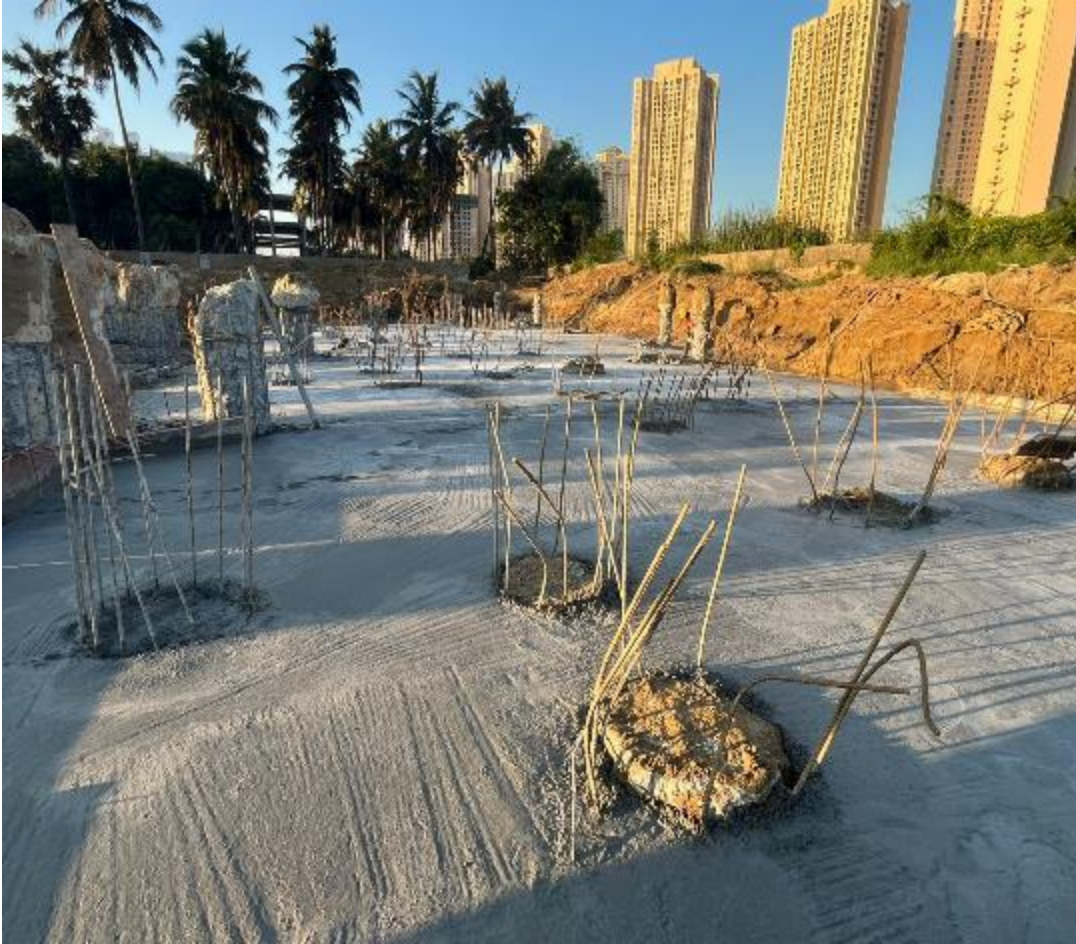
iHeart – Wing 1 PCC & Lift Pit Wall Reinforcement Work
