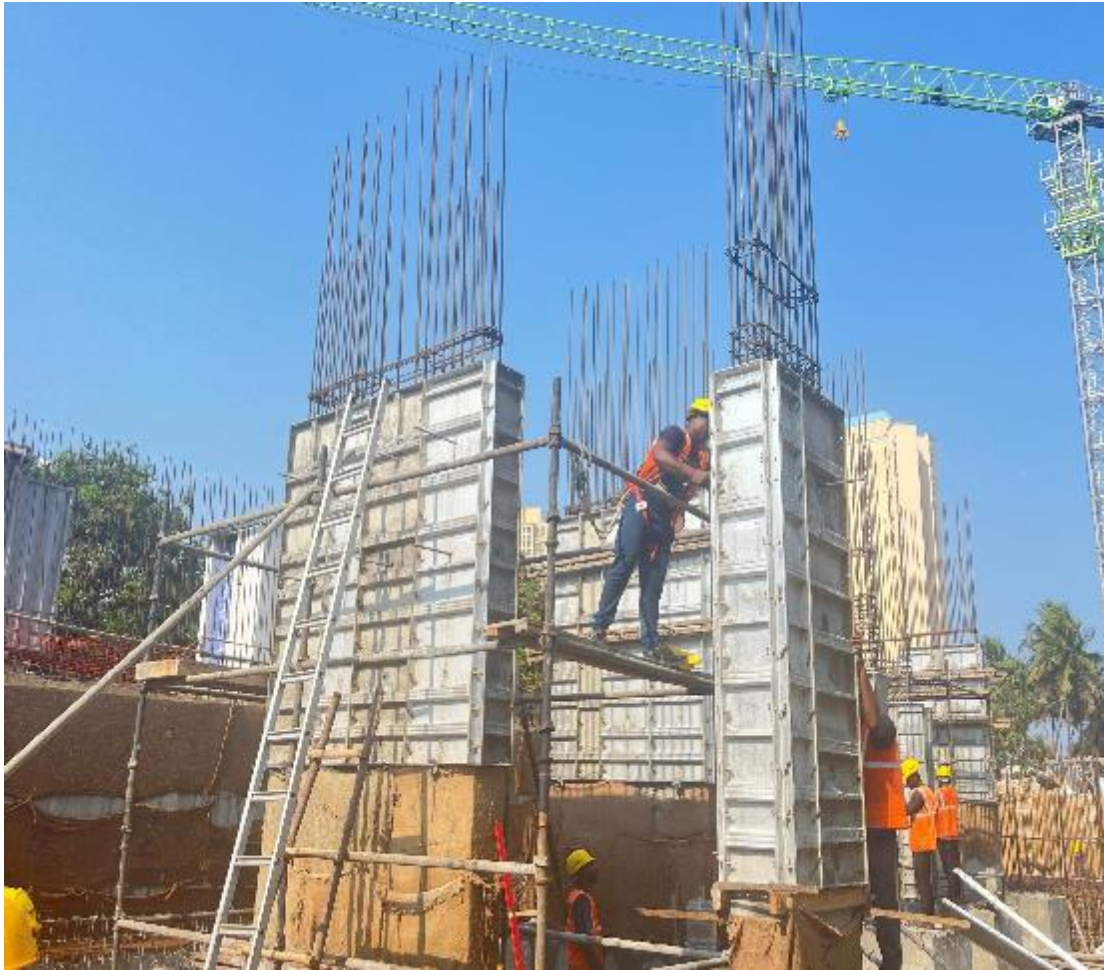
DRA iHeart – Wing 2 Column Shuttering Work
