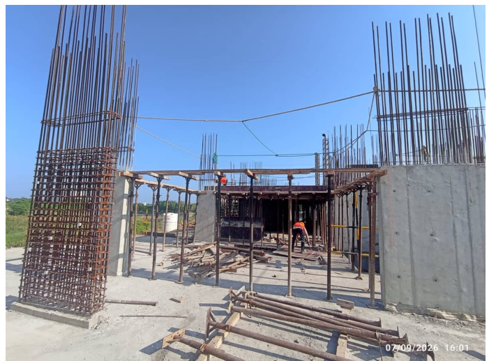
First Floor Slab Shuttering
