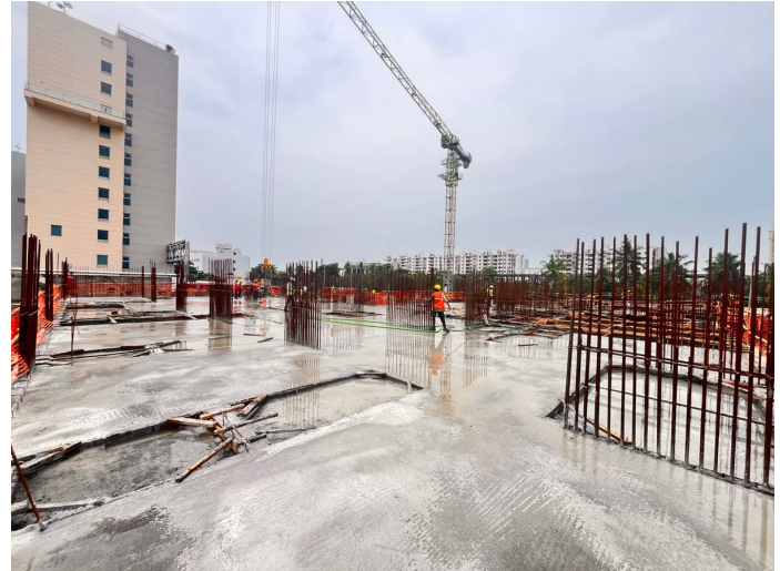
First Floor Slab Concrete
