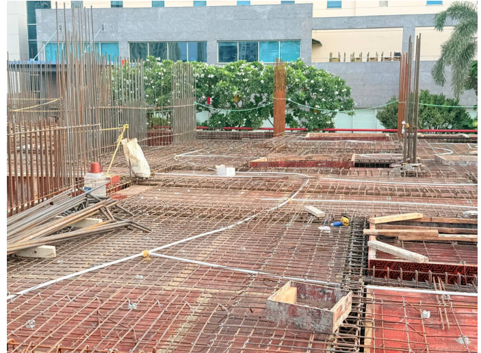
First Floor Slab Reinforcement
