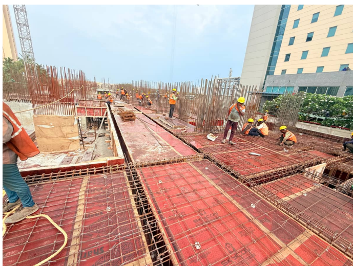
First Floor Slab Reinforcement
