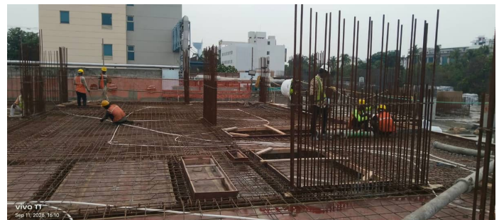
First Floor Slab Reinforcement
