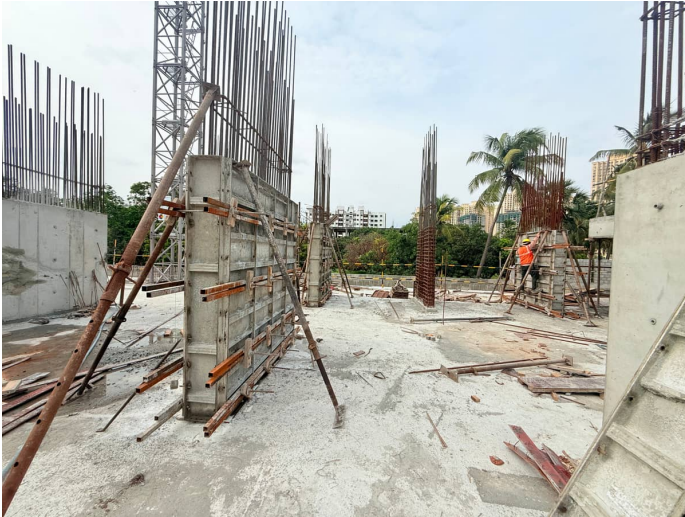
Column Reinforcement
