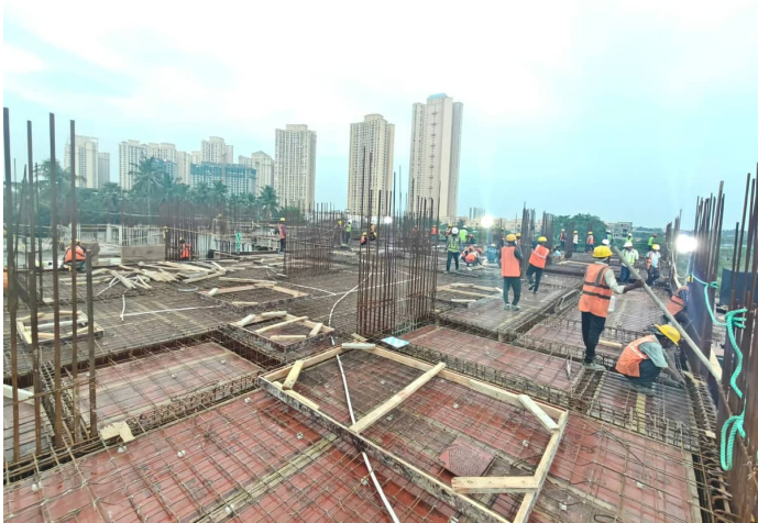
First Floor Slab Shuttering
