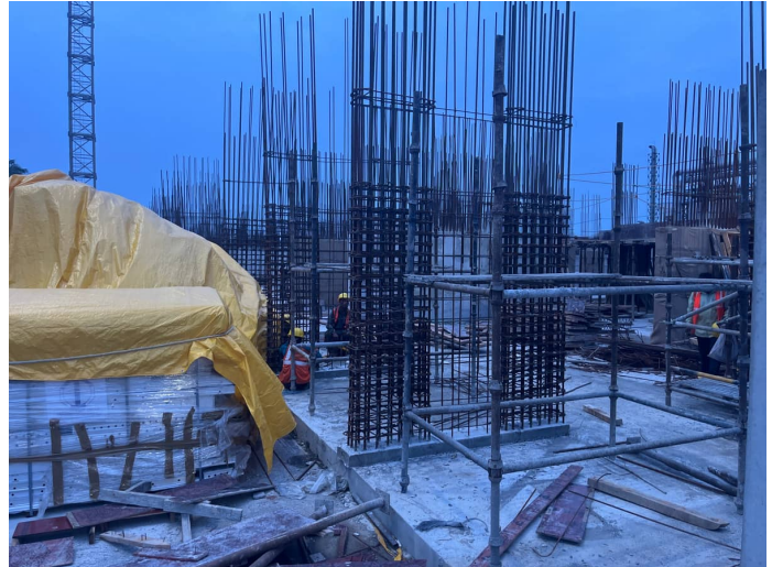
Column Reinforcement
