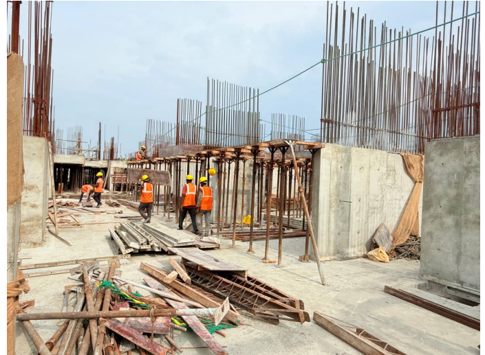
First Floor Slab Shuttering
