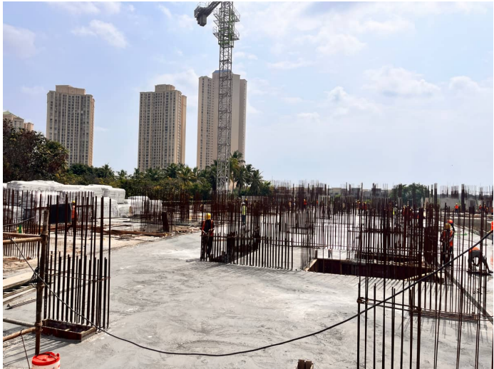
Stilt Floor Slab Concrete
