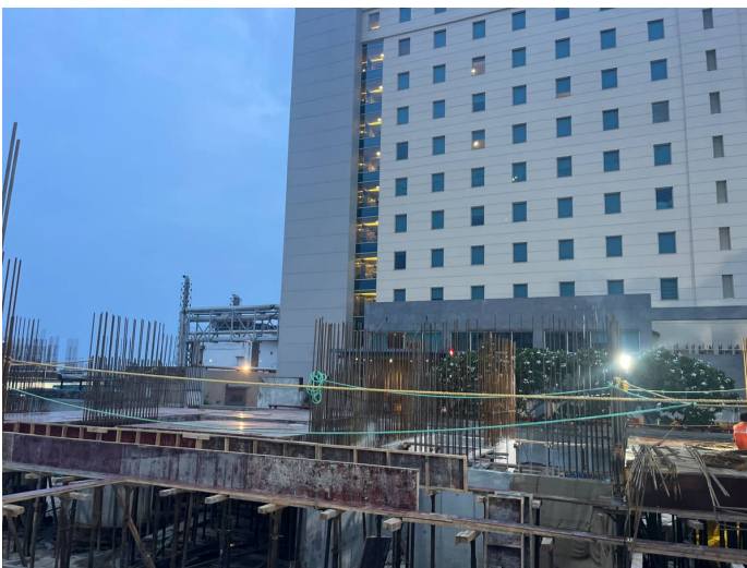
First Floor Slab Shuttering
