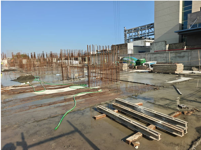
Stilt Floor Slab Concrete
