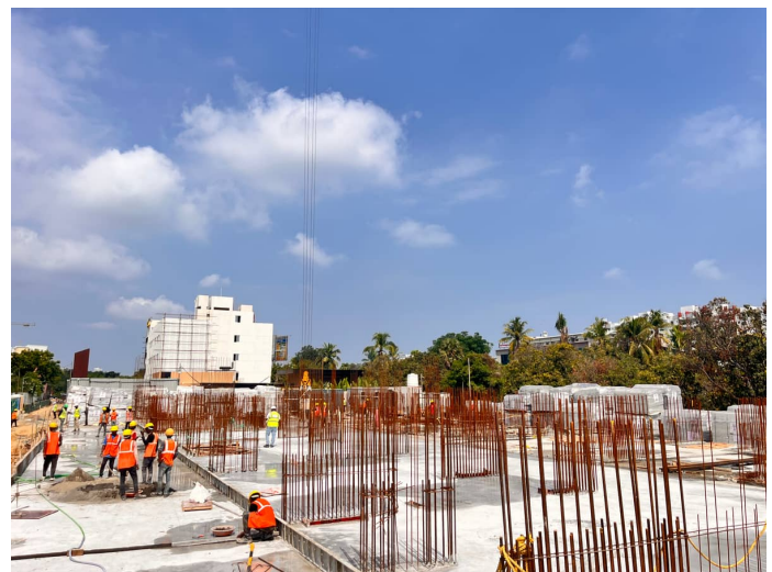
Column Reinforcement
