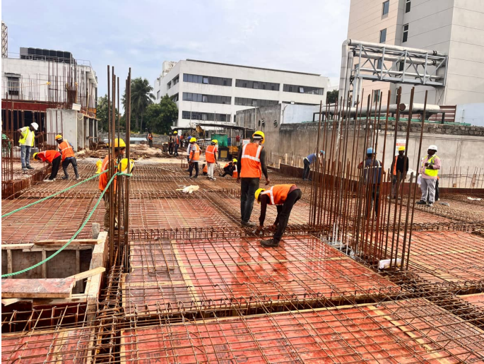
Stilt Floor Slab Shuttering
