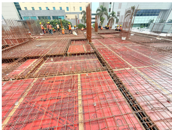
First Floor Slab Reinforcement
