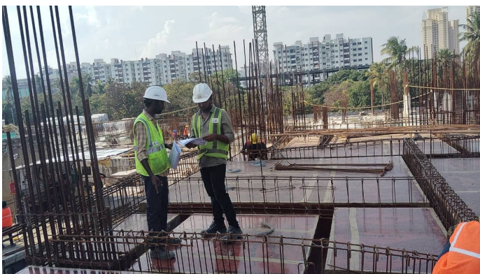
First Floor Slab Reinforcement
