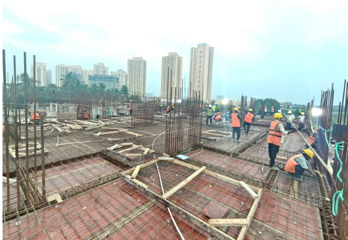
First Floor Slab Reinforcement
