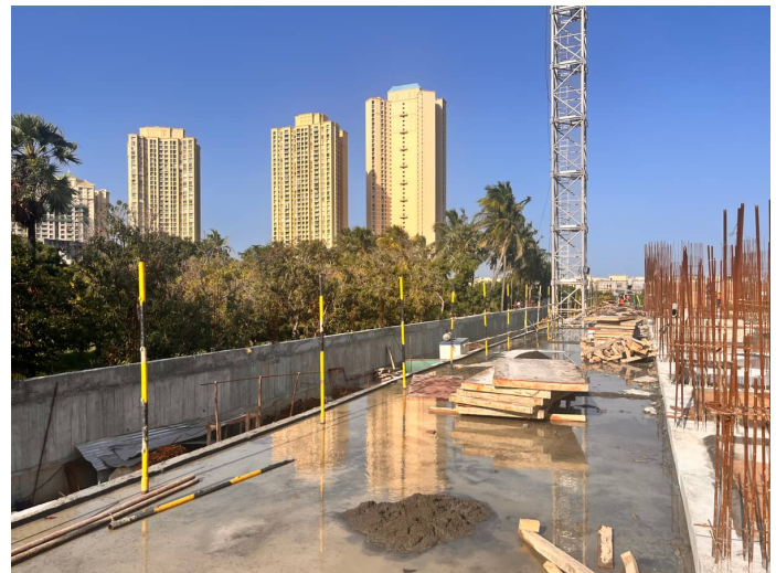
Stilt Floor Slab Concrete
