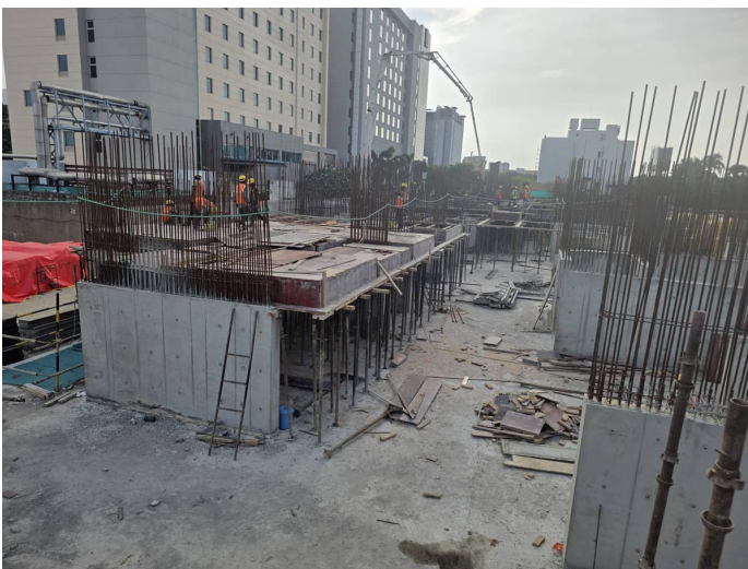
Column Reinforcement
