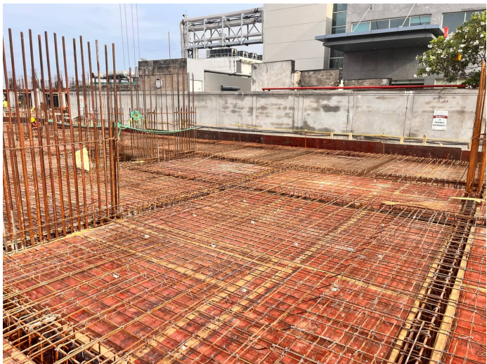
Stilt Floor Slab Shuttering
