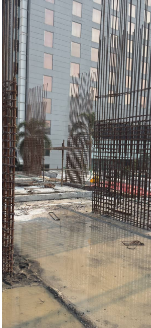
Column Reinforcement
