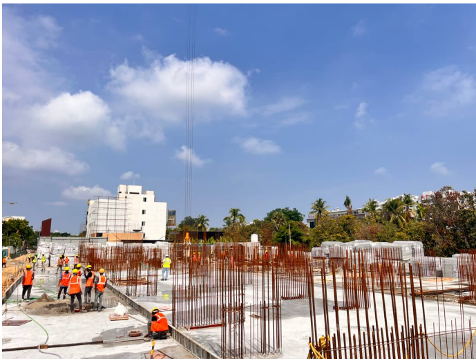
Stilt Floor Slab Shuttering
