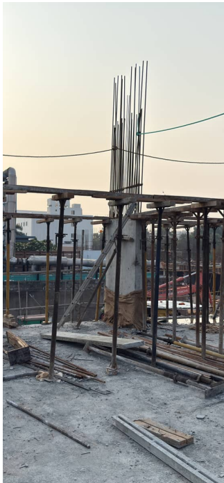
Second Floor Slab Shuttering
