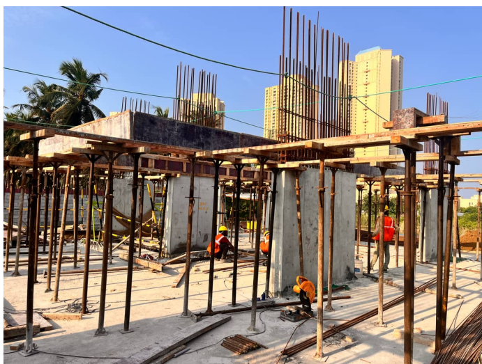
First Floor Slab Shuttering
