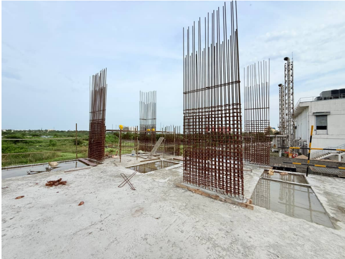
Column Reinforcement
