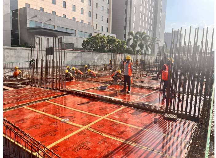
Stilt Floor Slab Shuttering
