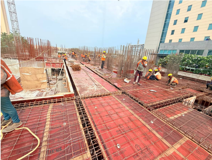
First Floor Slab Shuttering
