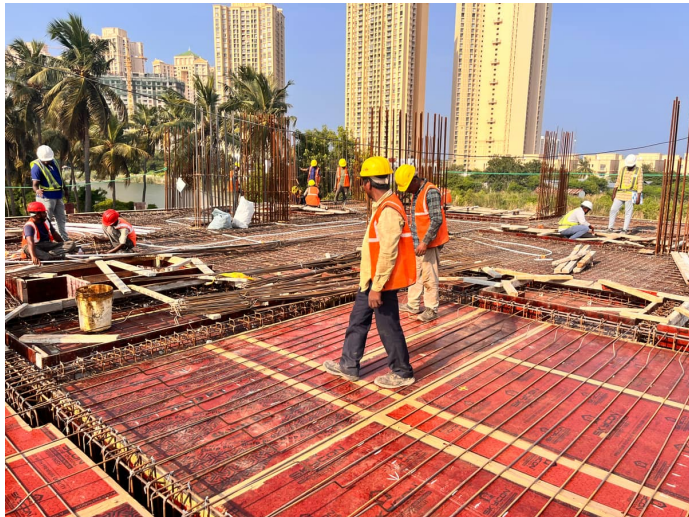
First Floor Slab Reinforcement
