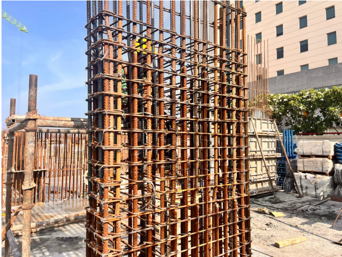
Column Reinforcement
