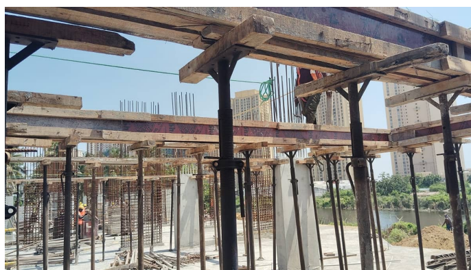
First Floor Slab Shuttering
