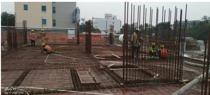
First Floor Slab Shuttering
