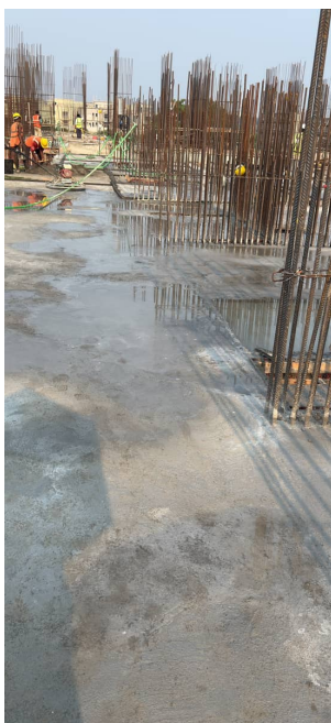
First Floor Slab Concrete
