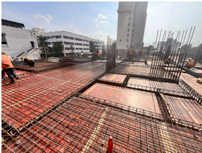
First Floor Slab Shuttering
