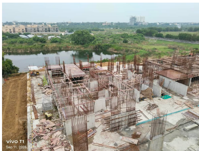
First Floor Slab Shuttering
