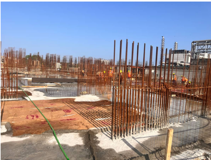
Stilt Floor Slab Concrete
