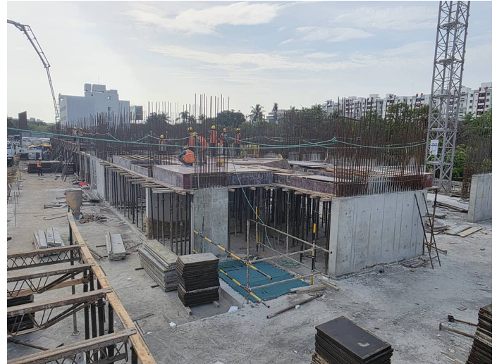
First Floor Slab Shuttering
