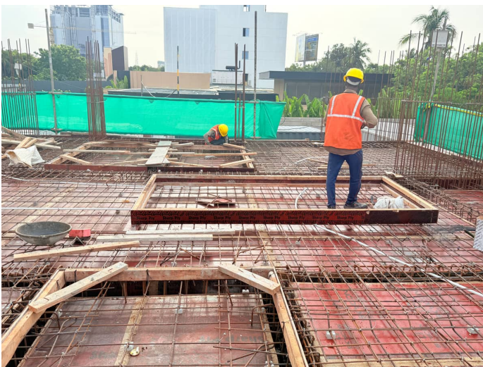
First Floor Slab Reinforcement
