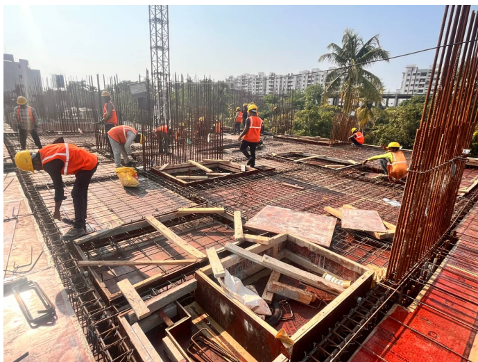
First Floor Slab Shuttering
