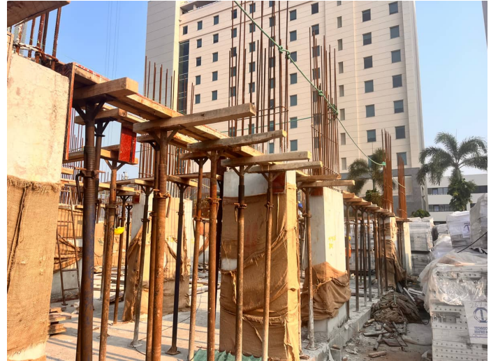
First Floor Slab Shuttering
