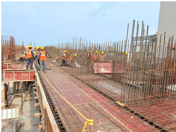
First Floor Slab Shuttering
