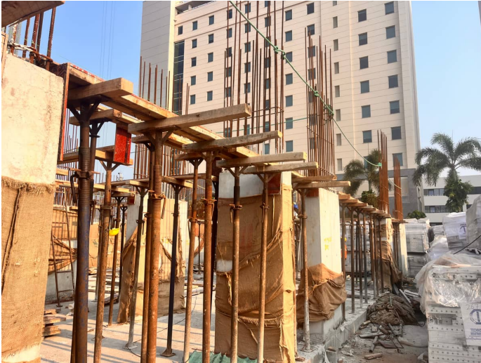
First Floor Slab Shuttering
