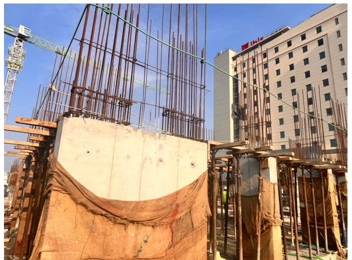
First Floor Slab Shuttering
