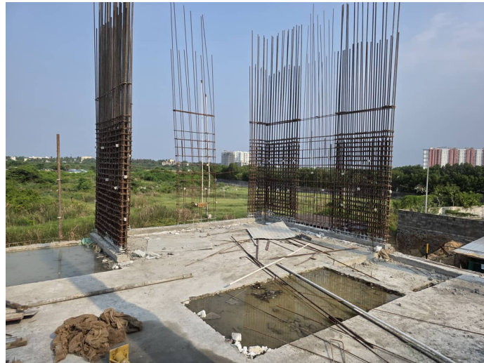
Column Reinforcement
