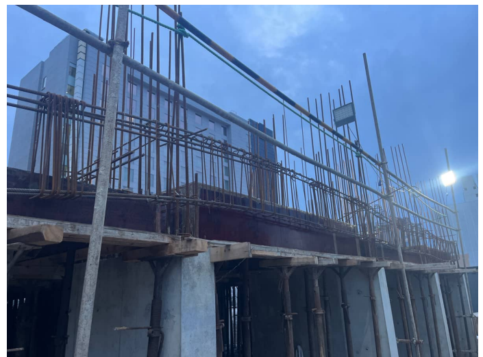
First Floor Slab Reinforcement
