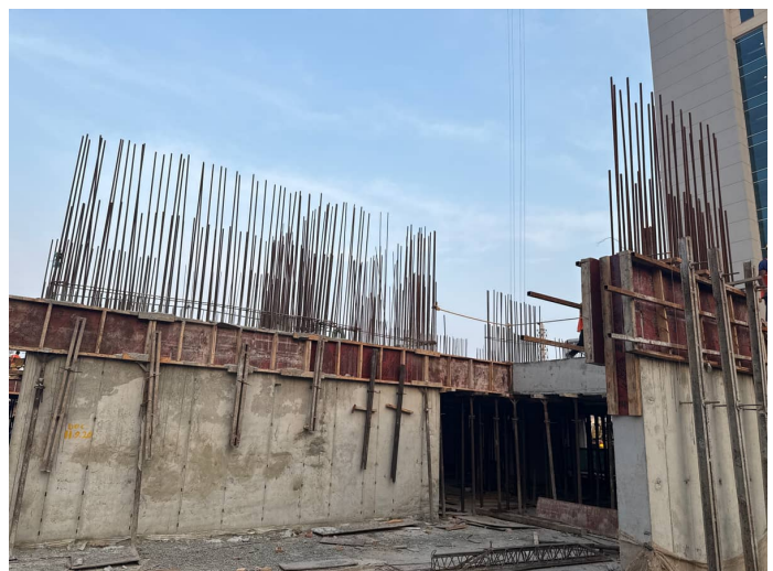
First Floor Slab Shuttering
