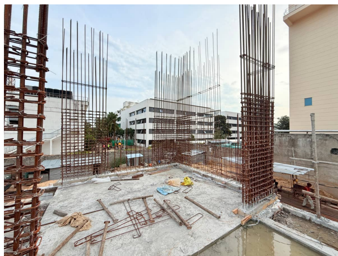
Column Reinforcement
