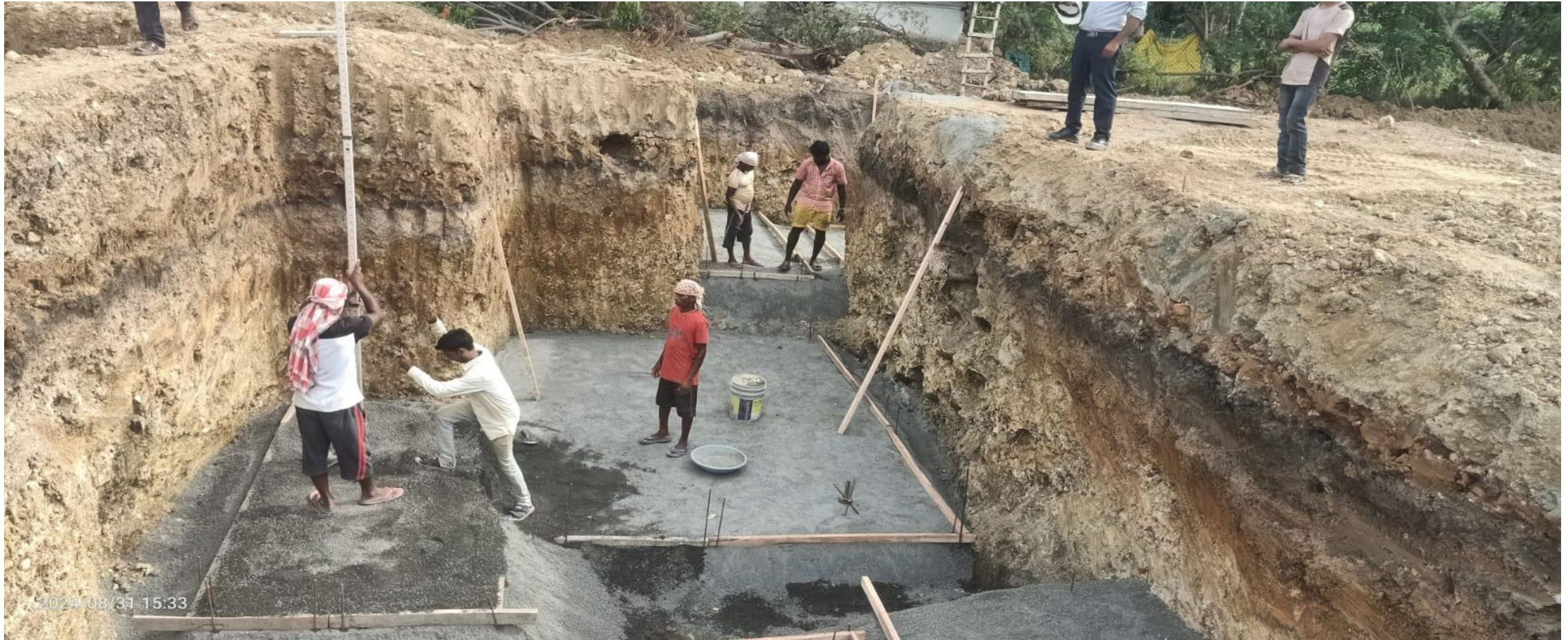
Villa No.08 Footing Quarry Dust Filling Work
