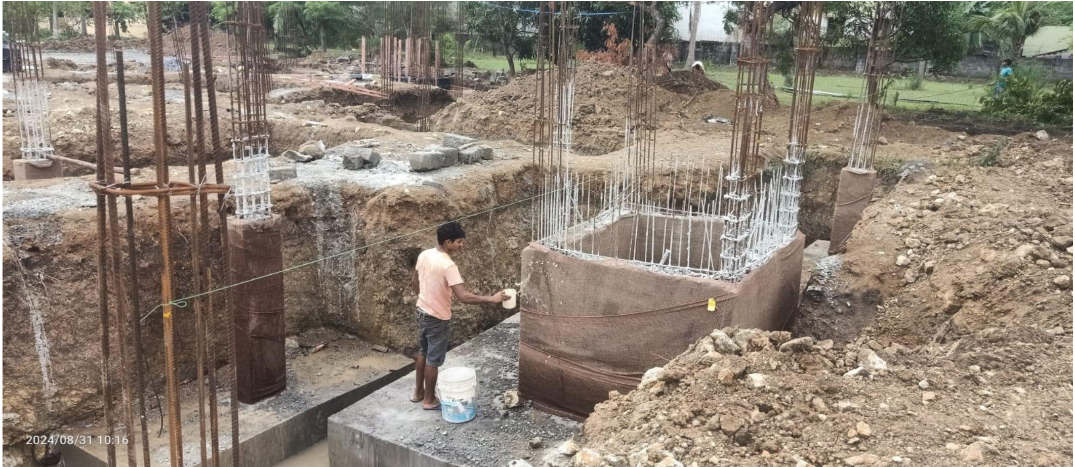
Villa No.06 Lift wall concrete curing work
