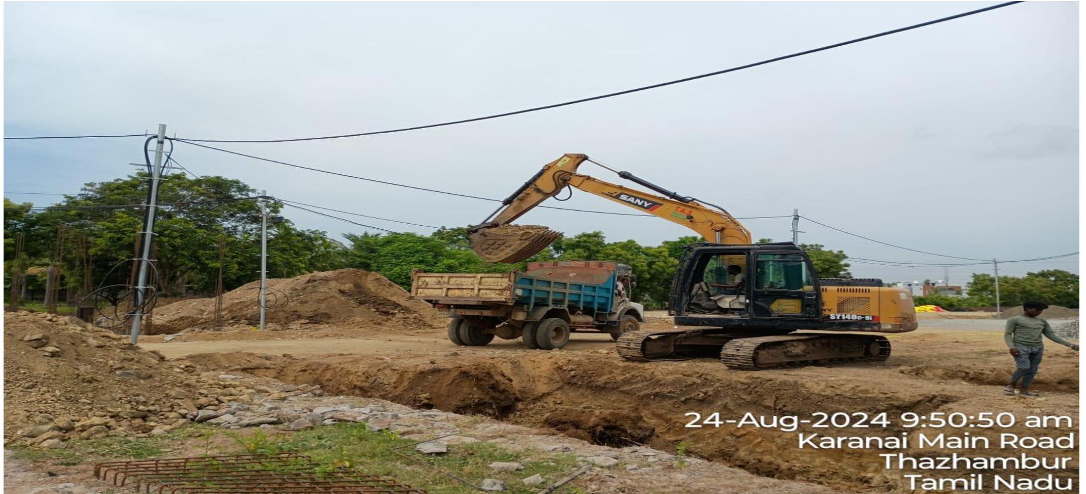
Villa No.16 Footing Earthwork Excavation work
