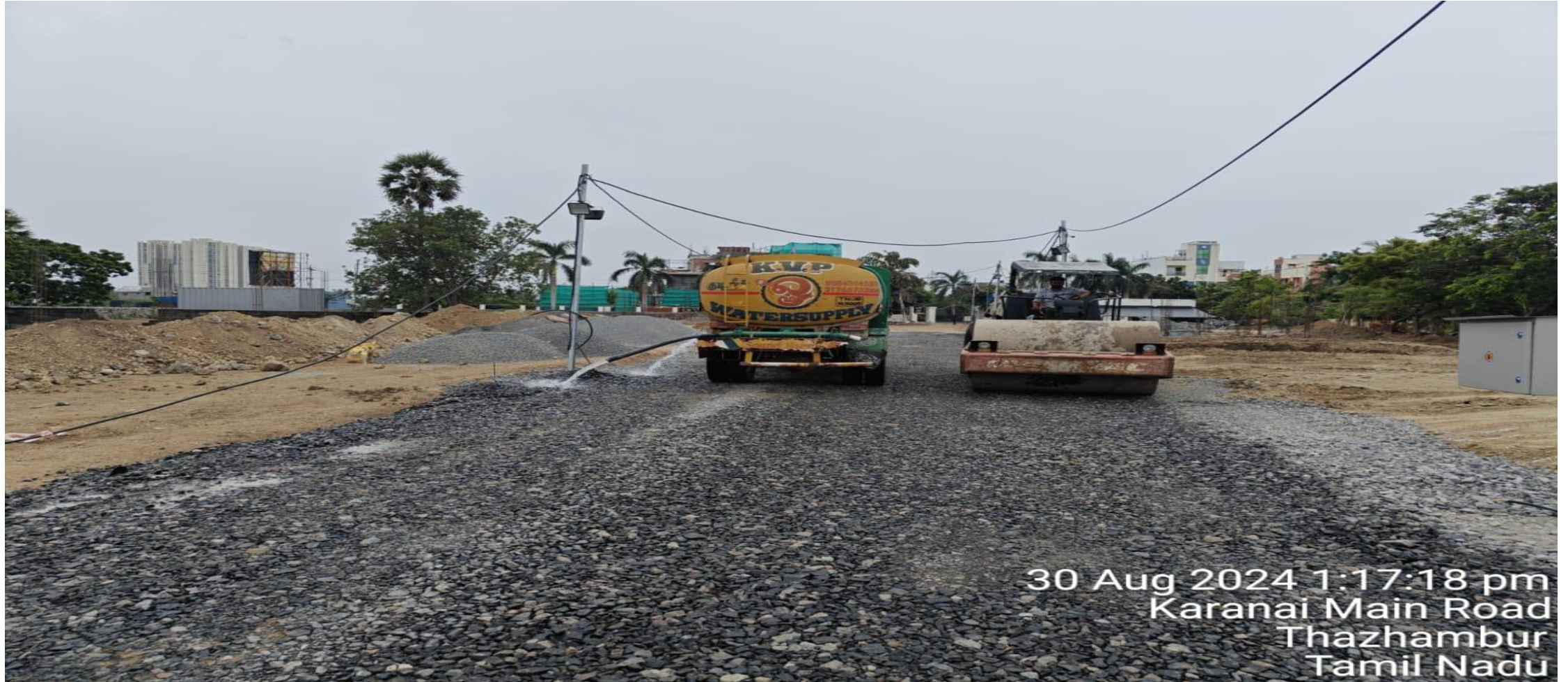
Road GSB Rolling & Compaction work
