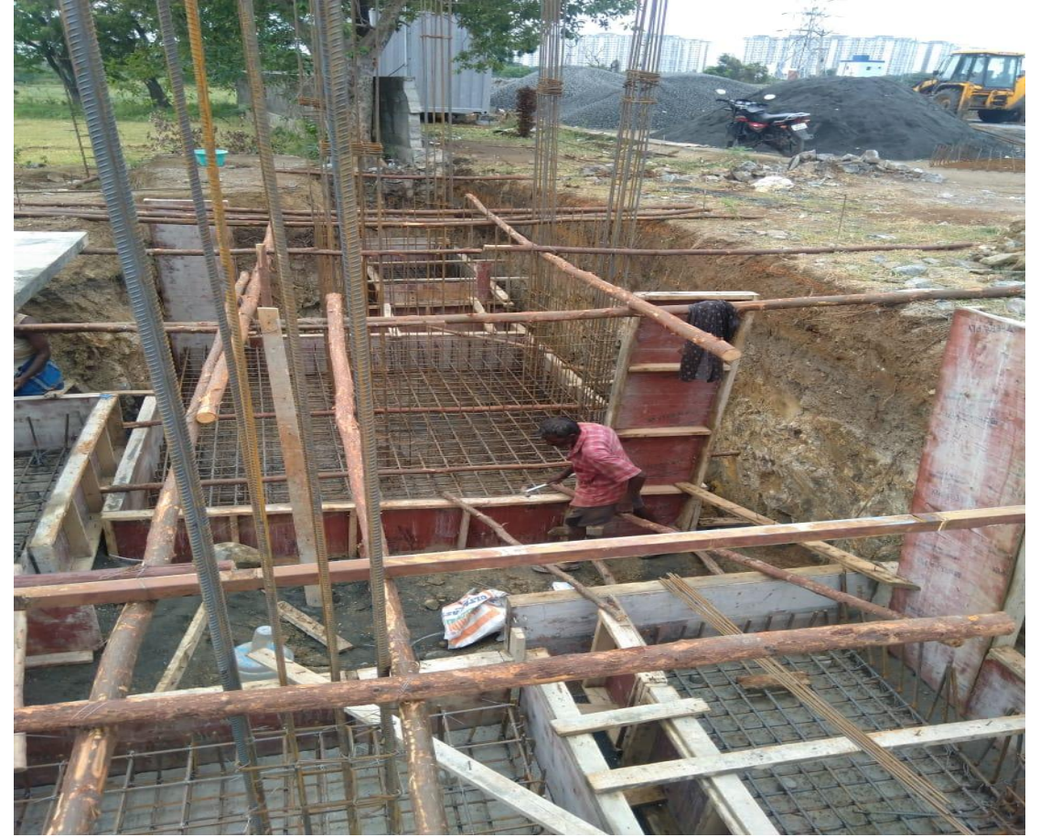
Villa No.16 Footing & Column Reinforcement and Shuttering work
