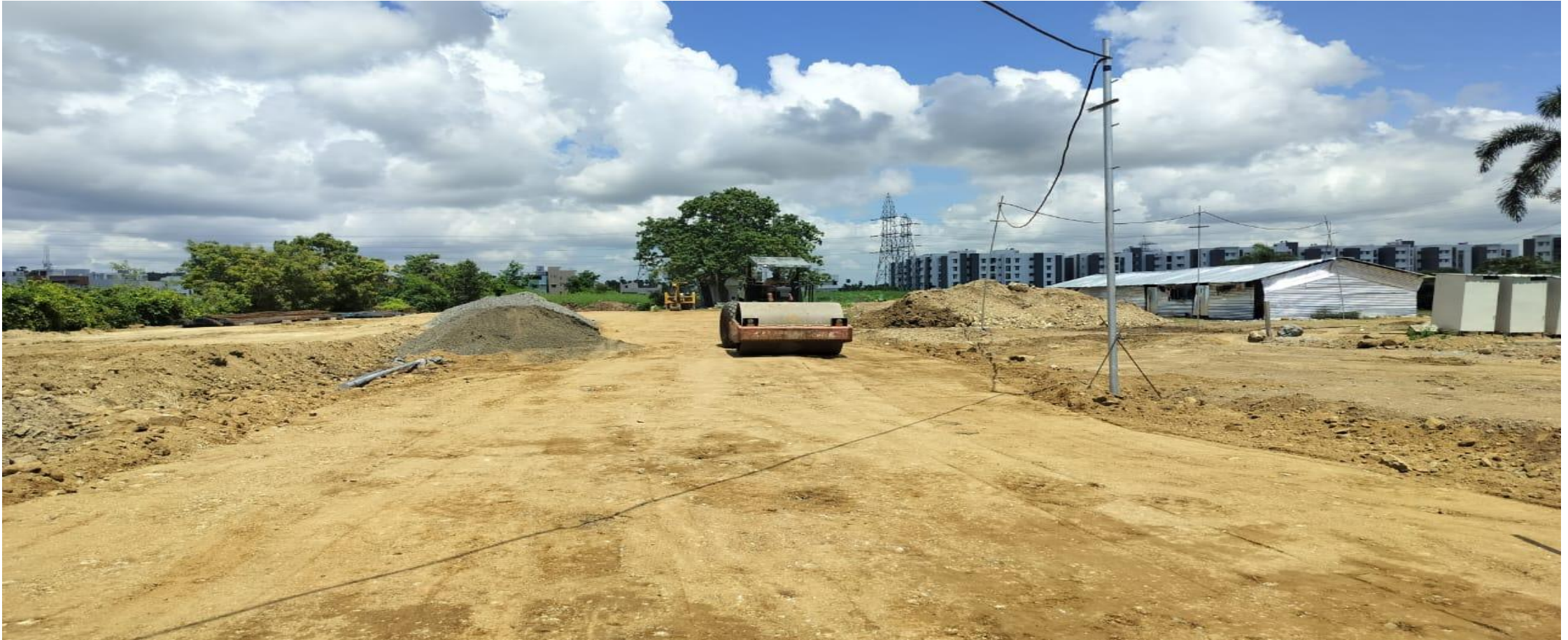
Road Hill Earth Compaction work
