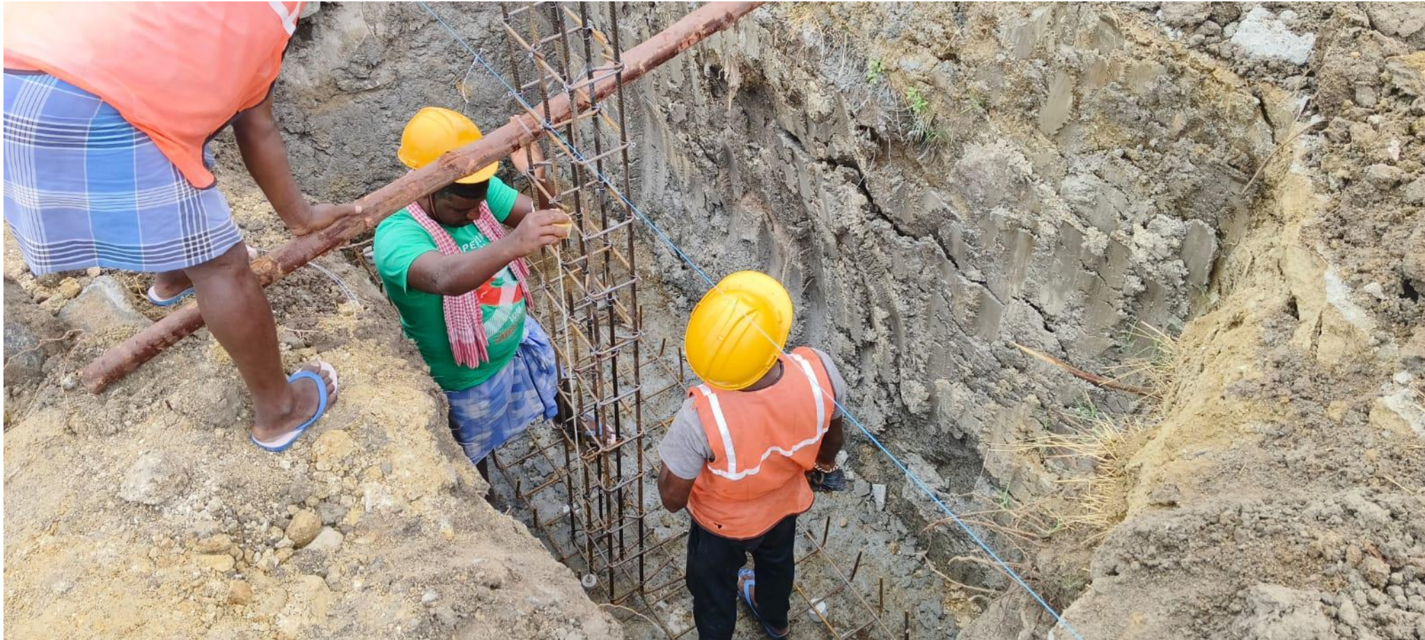
Compound wall Footing & Column Steel Reinforcement work
