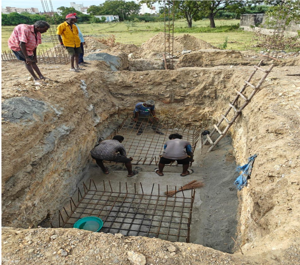
Villa No.16 Footing & Column Reinforcement and Shuttering work
