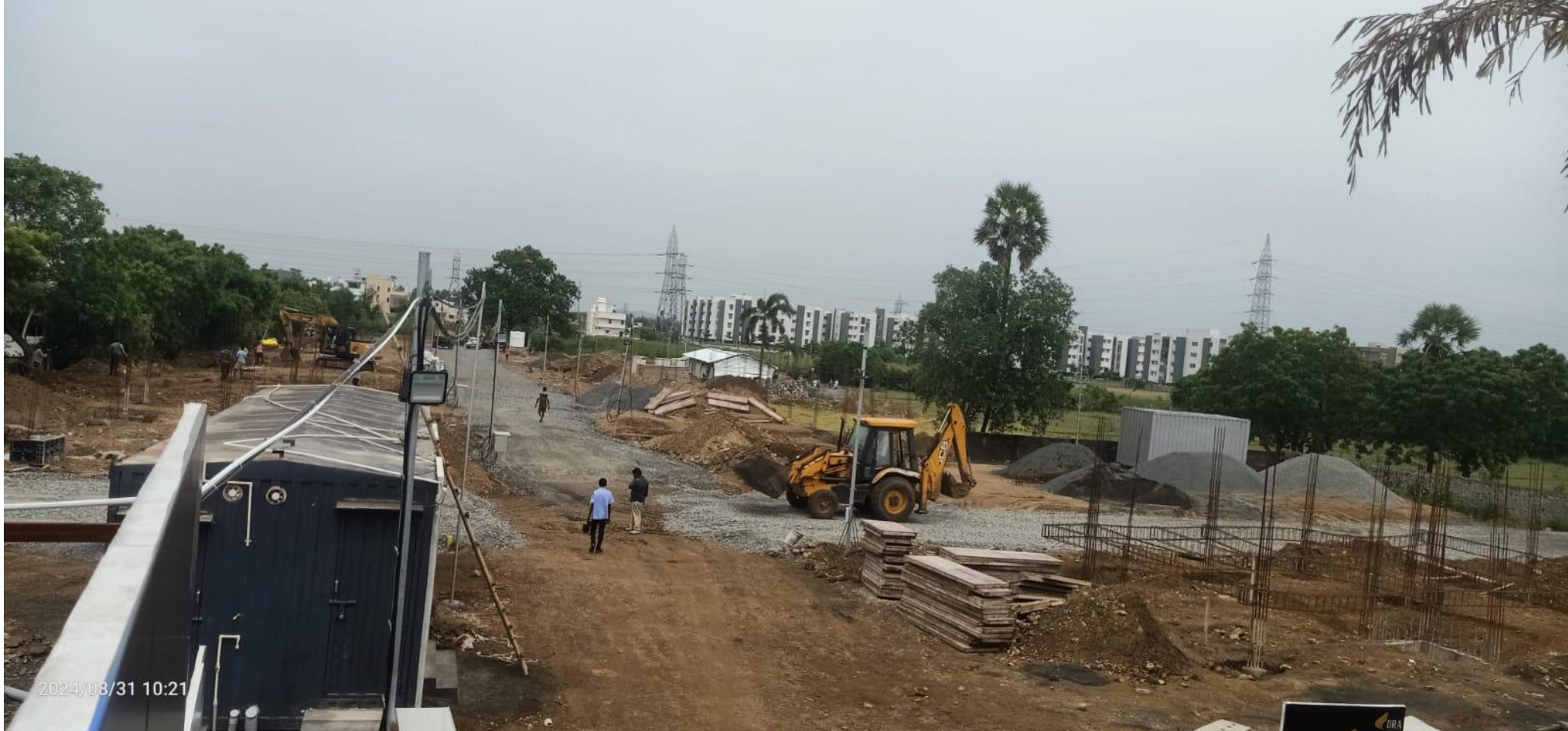
ROAD GSB FILLING WORK
