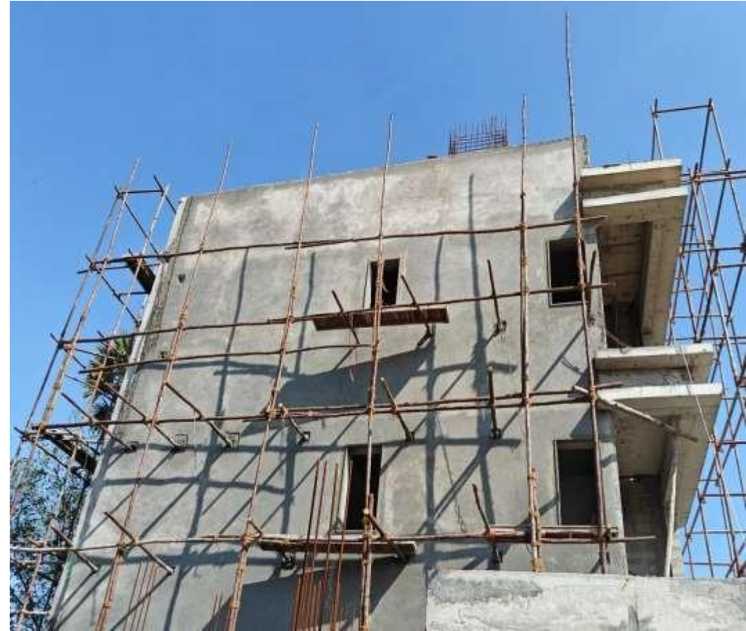
Villa no 16 – External plastering work in progress
