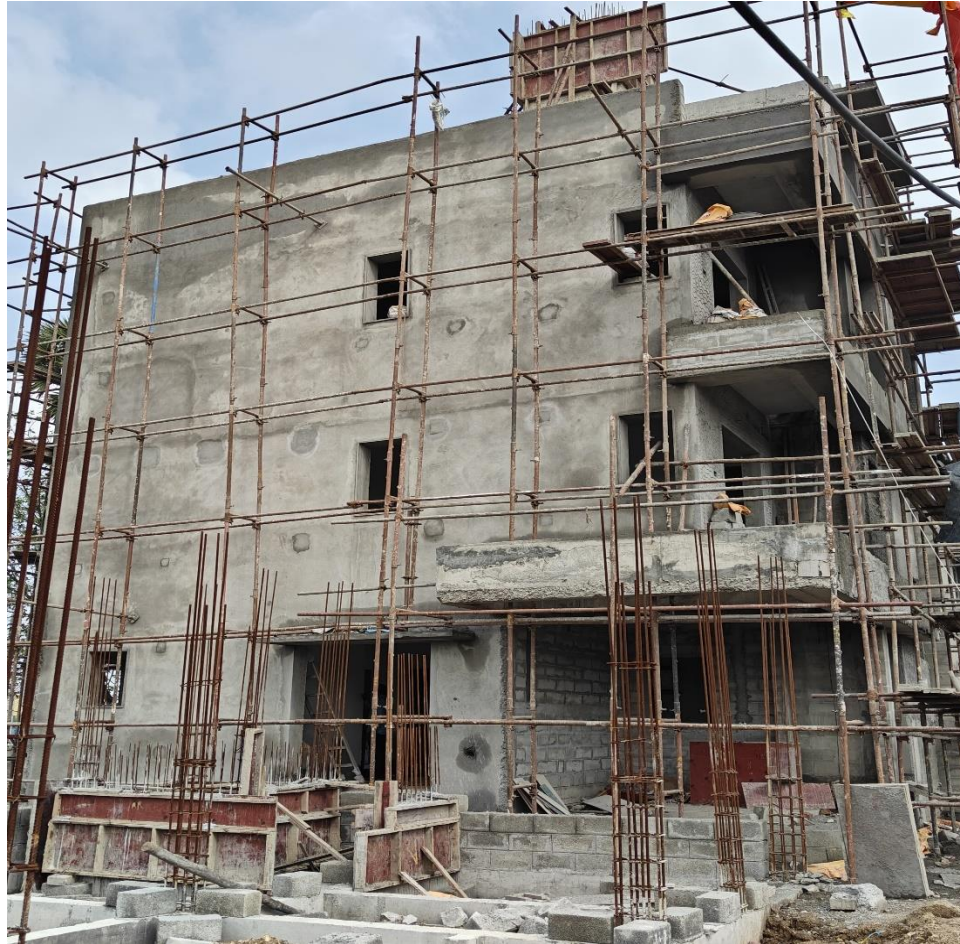
Villa no 16 – External plastering work in progress
