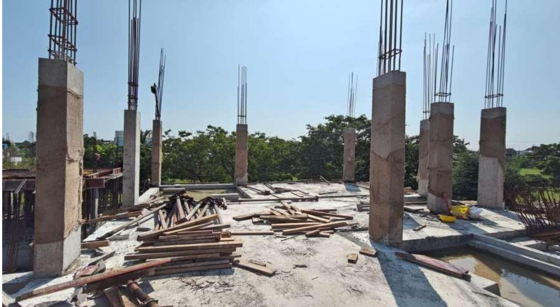
Villa No 6 – First Floor Column concreting work completed
