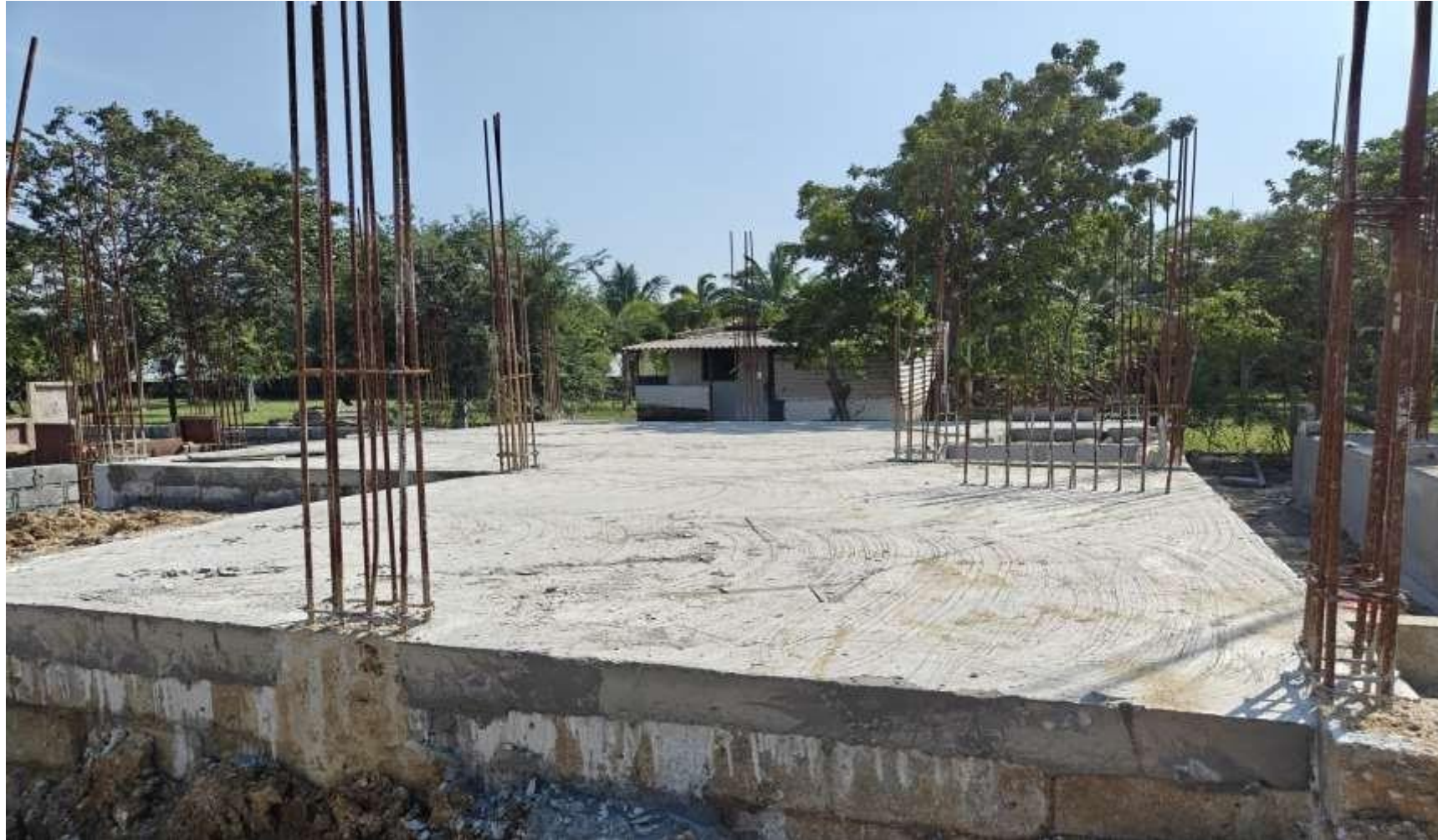
VillaNo 09 – GF Flooring PCC work completed
