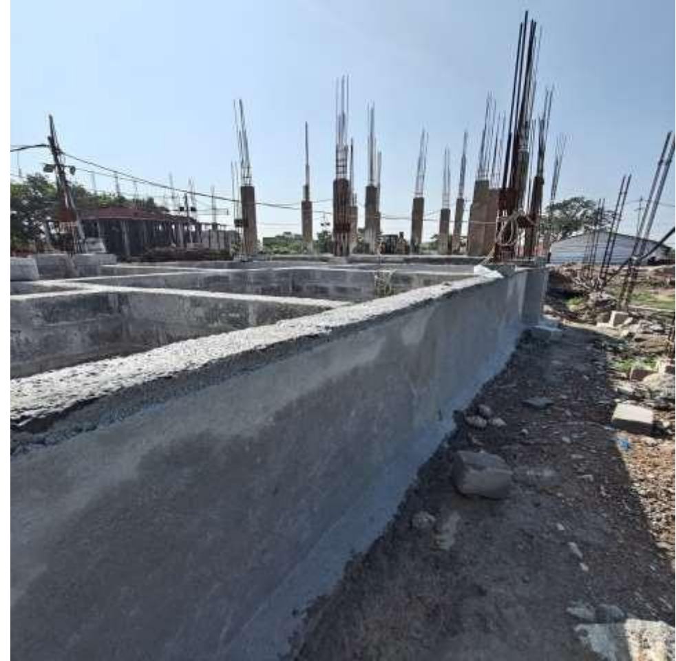
Villa No 05 & 13 DPC Protection Plastering work completed
