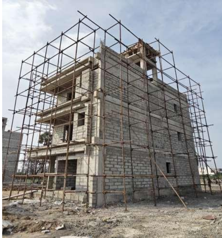
Villa no 20: Scaffolding fixing work completed
