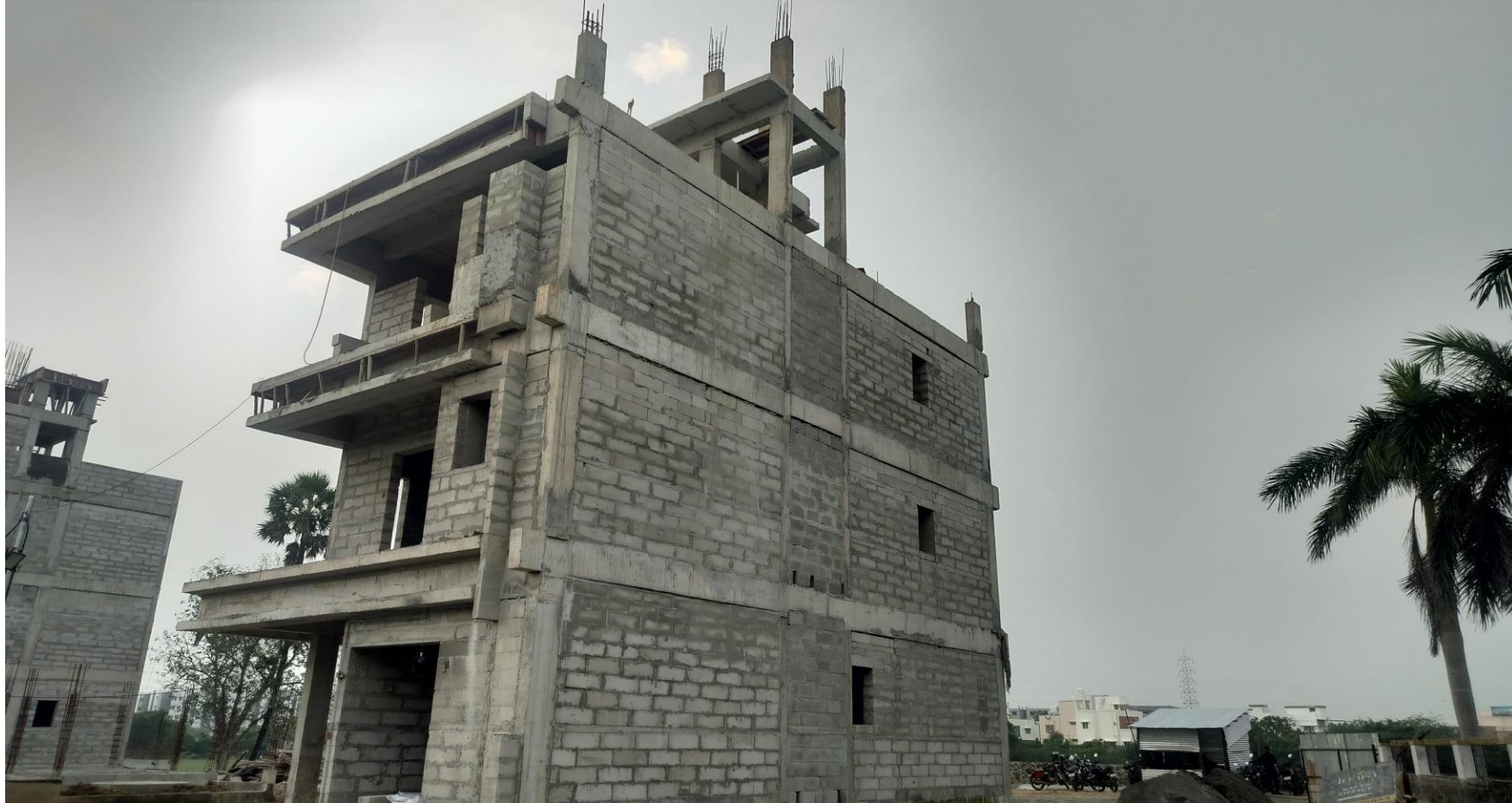
Villa no 20 South East corner View
