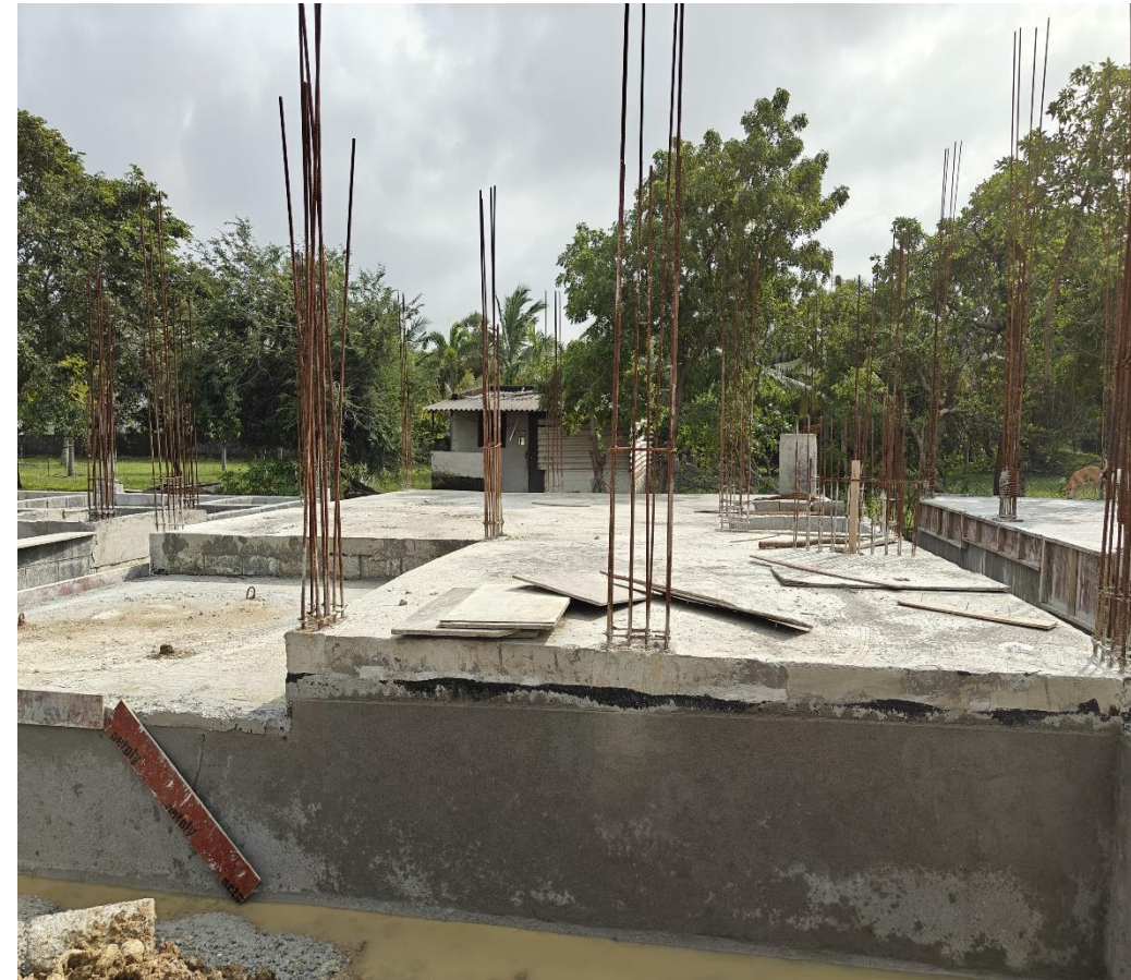
VillaNo 09 , 10 – GF Floor PCC work completed
