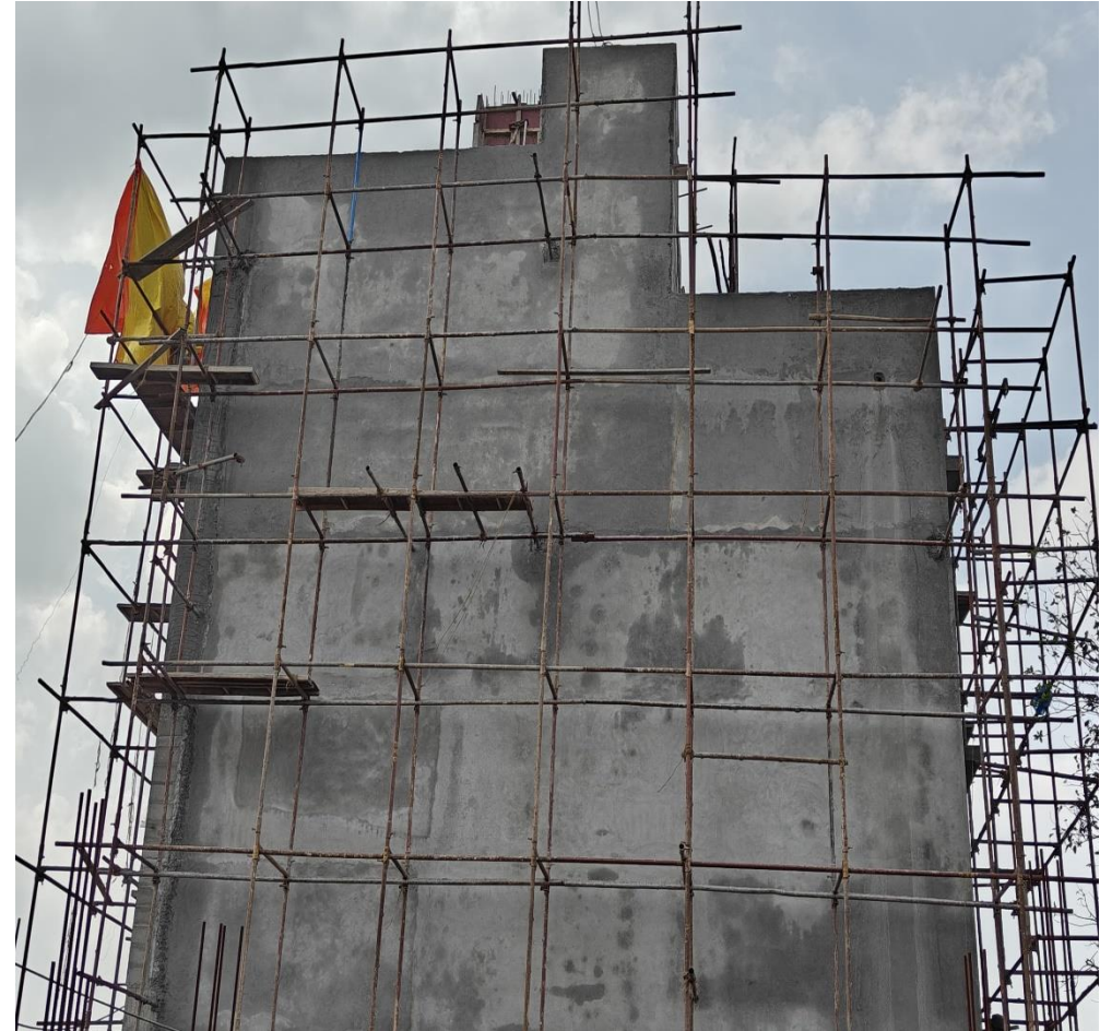
Villa no 16 – External plastering work in progress
