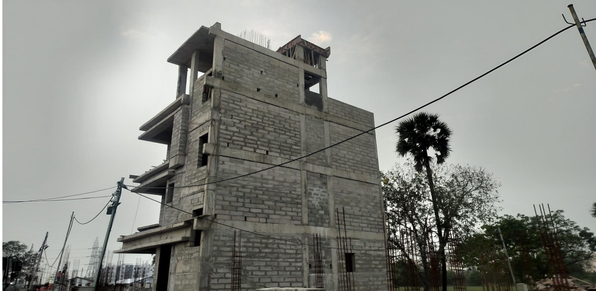
Villa no 16 – South East Corner View
