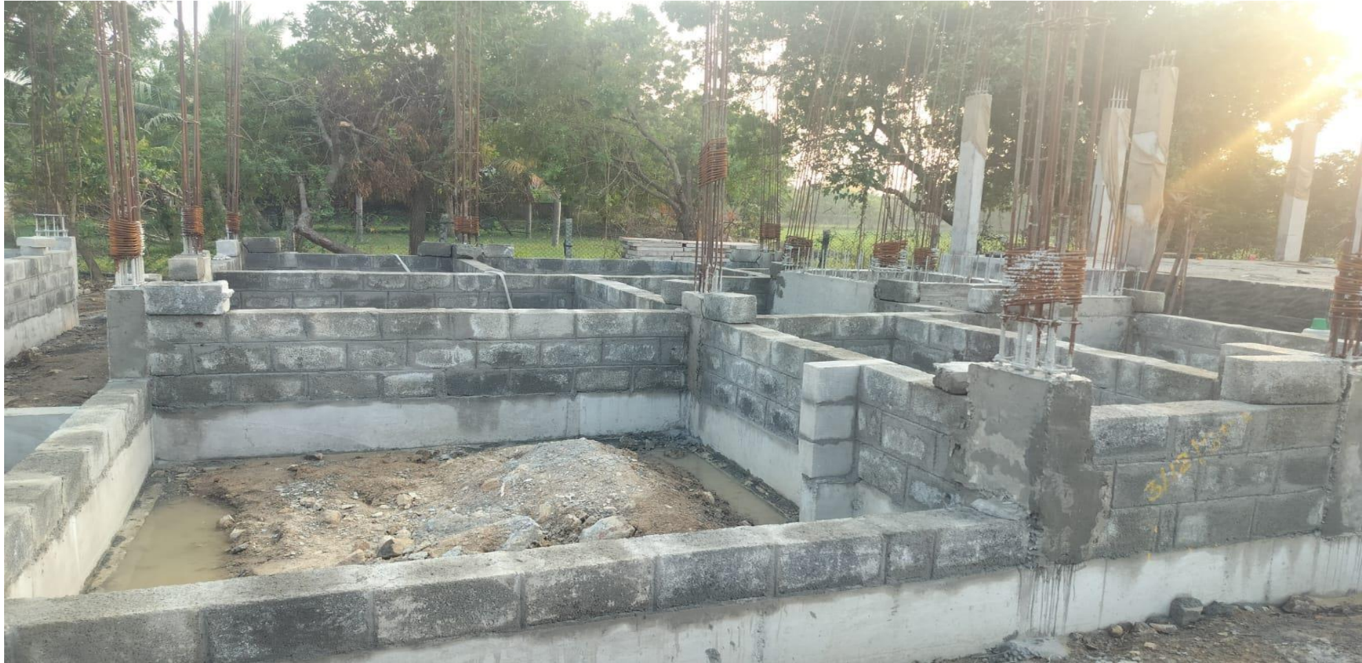
Villa No 10 – Above Plinth Beam Block Work in Progress
