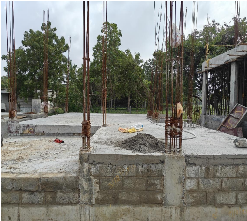
VillaNo 09 , 10 – GF Floor PCC work completed
