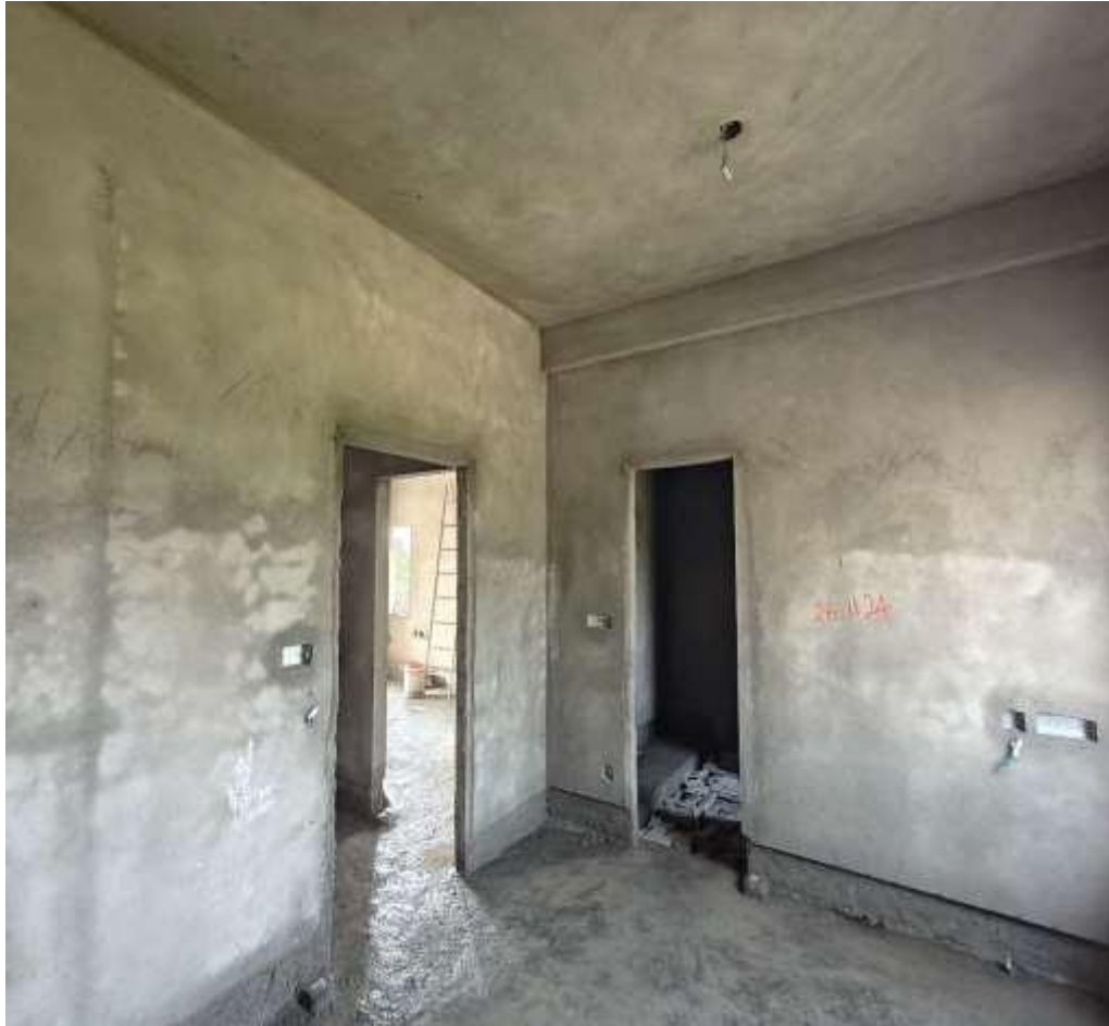
Villa No 16 – First Floor Internal wall Plastering work completed
