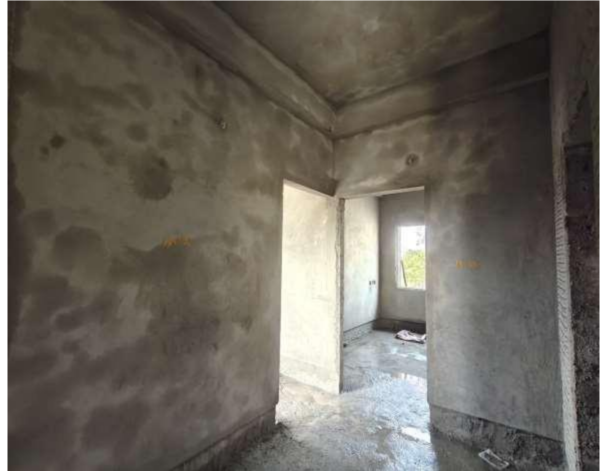
Villa No 16 – First Floor Internal wall Plastering work completed
