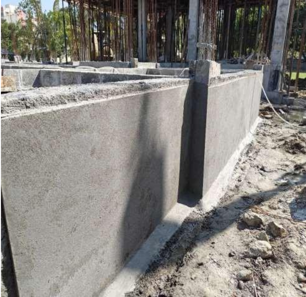
Villa No 05 & 13 DPC Protection Plastering work completed
