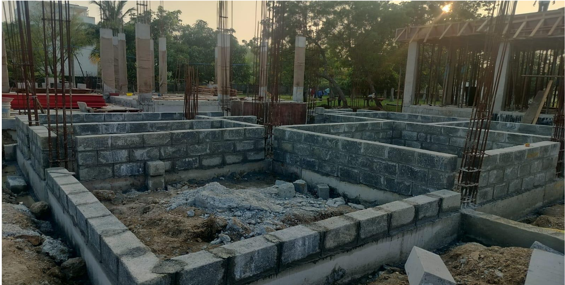
Villa No 5 – Above Plinth Beam Block Work in Progress
