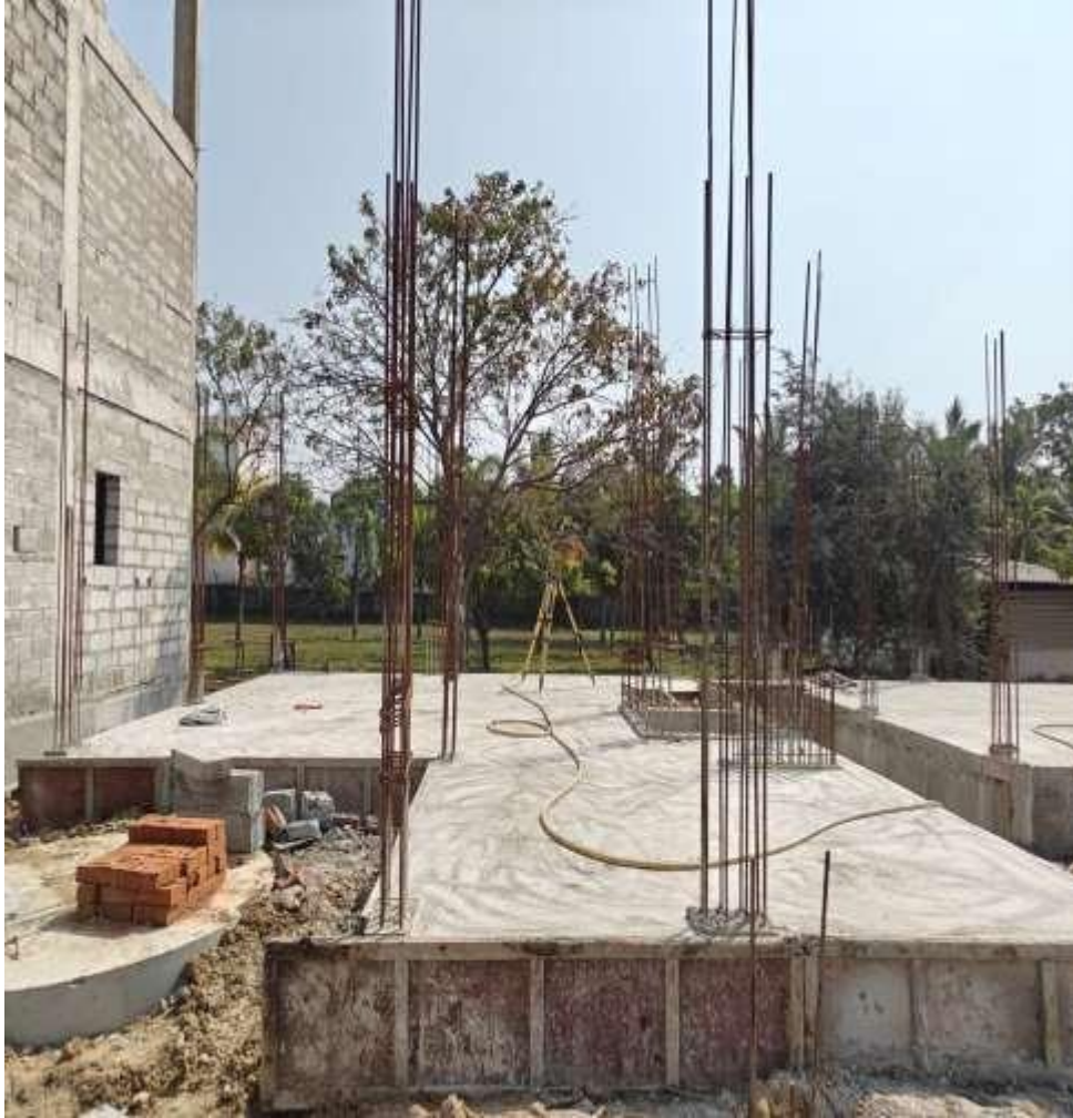
Villa No 7, 8 – GF Flooring PCC Pouring work completed
