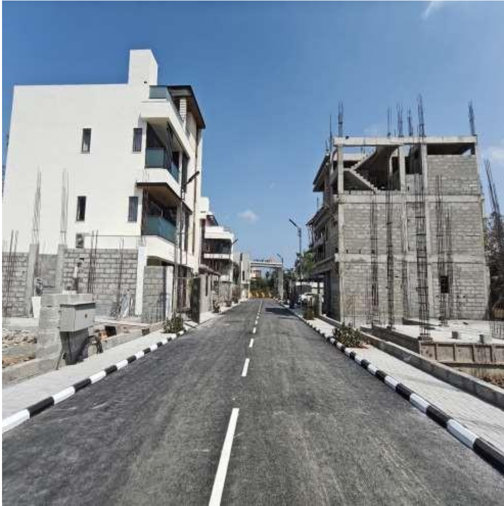
Internal Road DBM course Laying work completed
