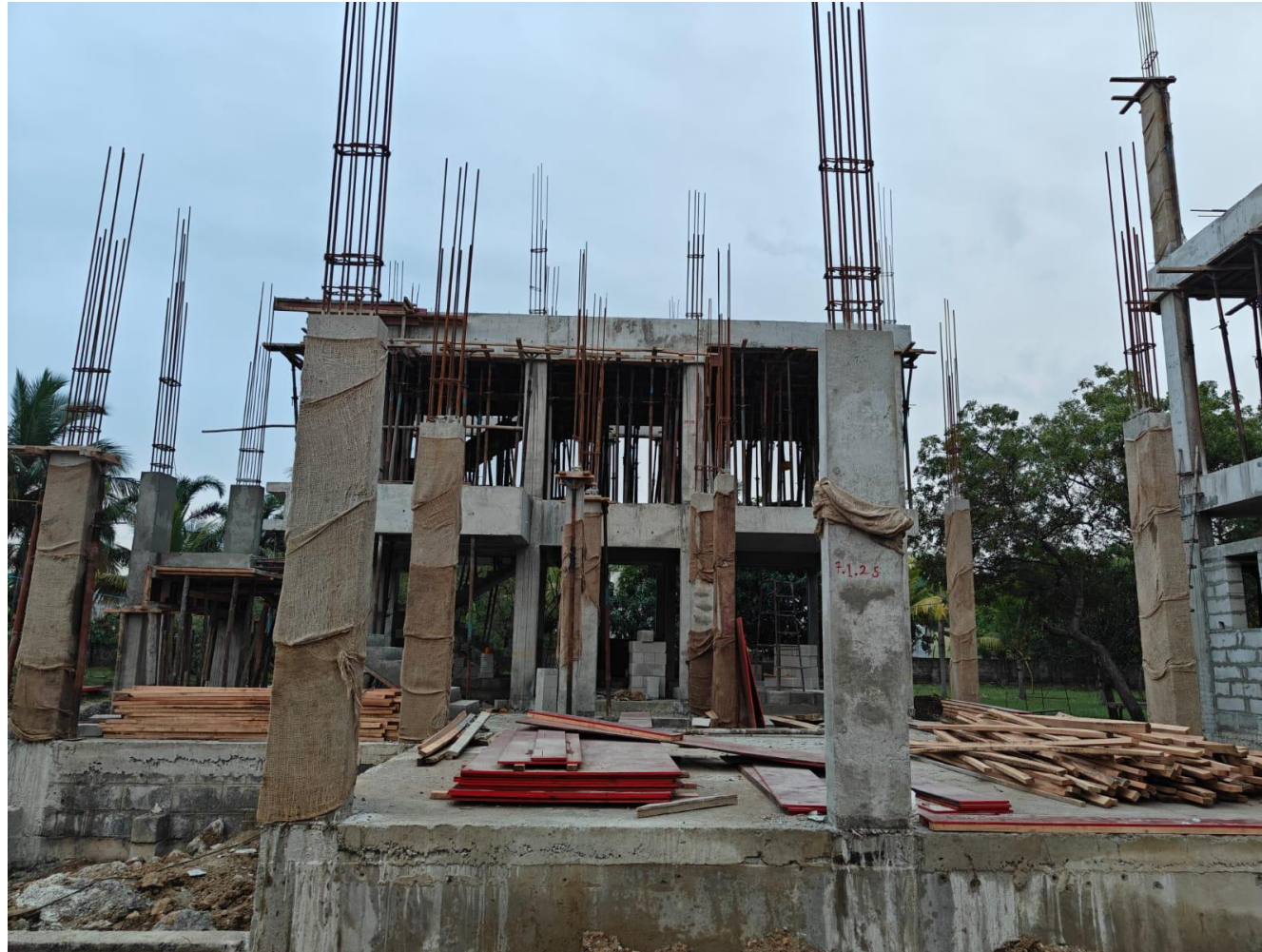
Villa No 5 – Ground Floor Column Concrete work Completed
