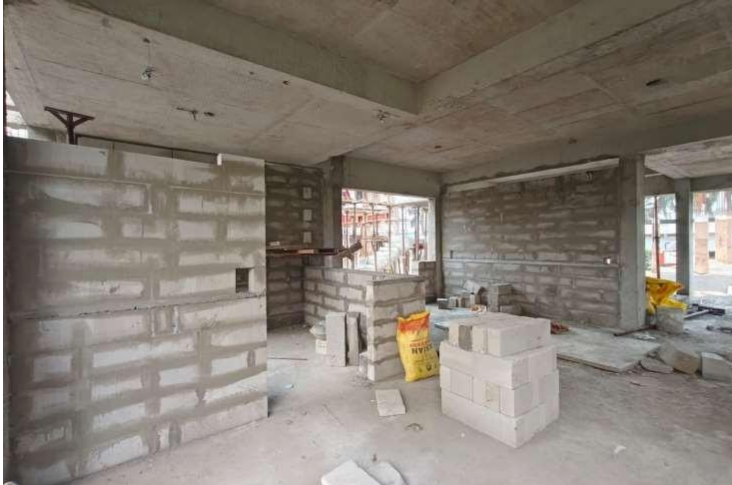
VillaNo 4 – Ground Floor Blockwork in progress
