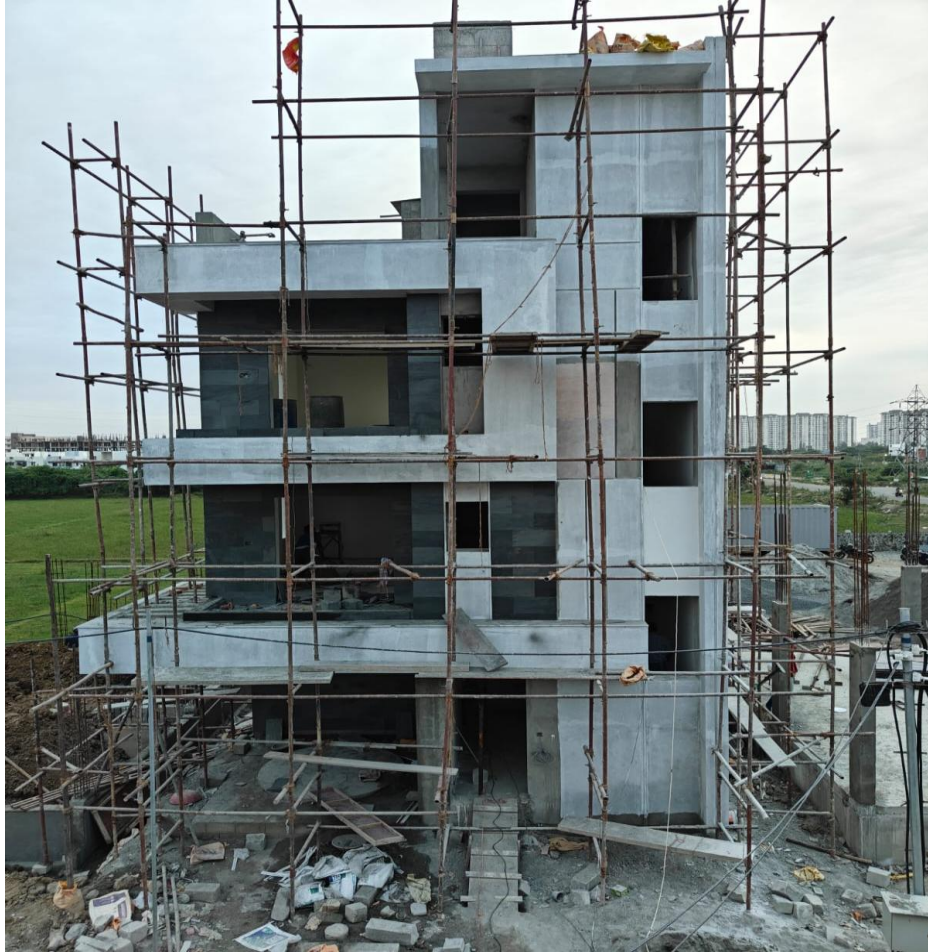
Villa no 16 – External Wall Bubble Texture and Painting work in Progress
