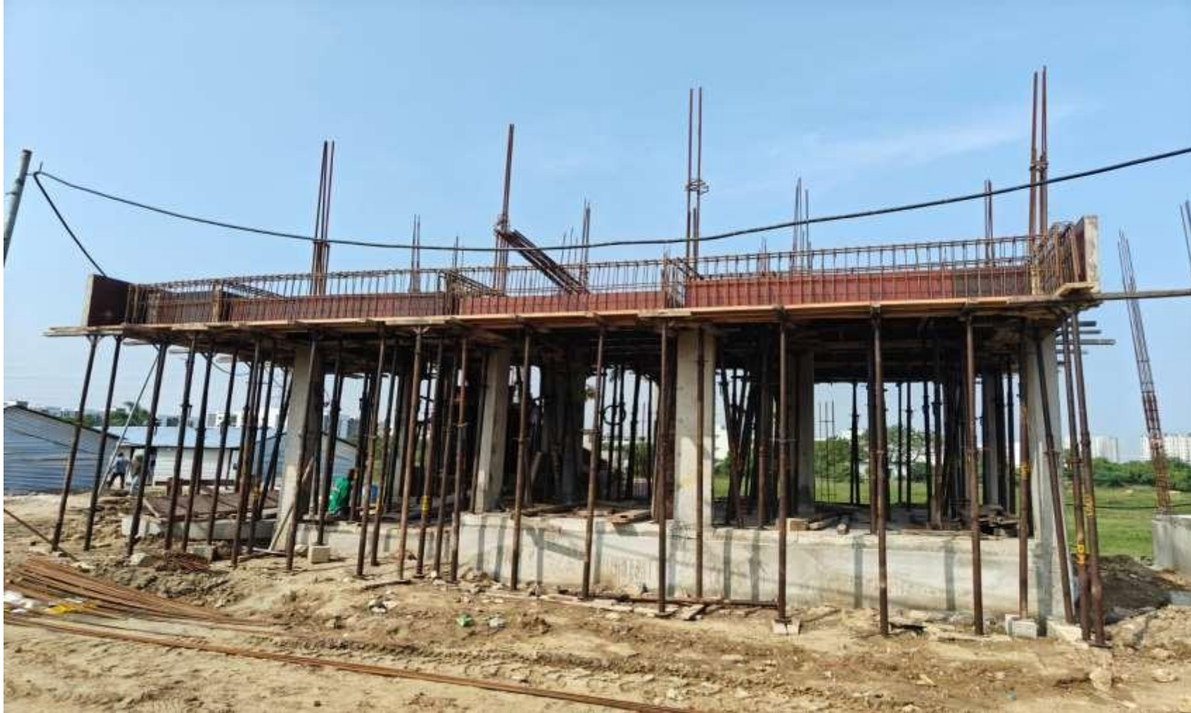
VillaNo 12 – GF Roof Slab Reinforcement work in progress
