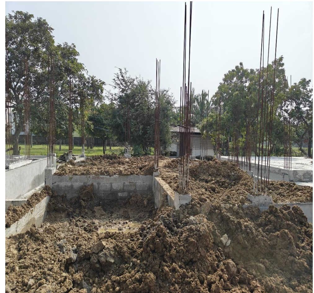
Villa no 07 , 08 – Basement Soil Backfilling work in progress
