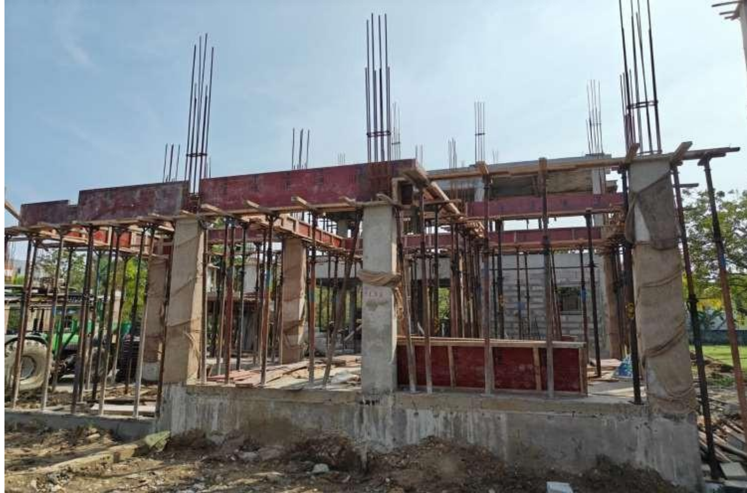
VillaNo 5 – Ground Floor Roof Slab Shuttering work in progress
