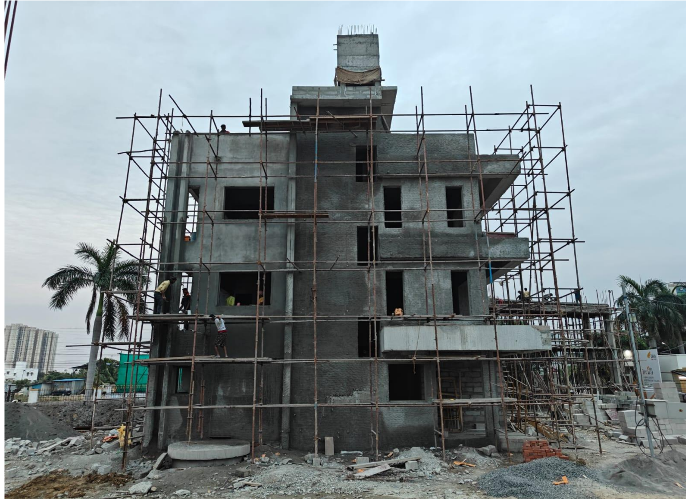
Villa No 20 – External wall plastering work in progress
