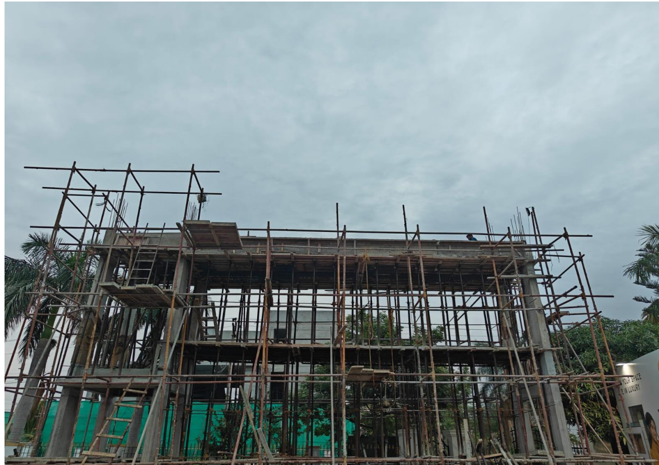
Entrance Arch Slab Concrete Completed
