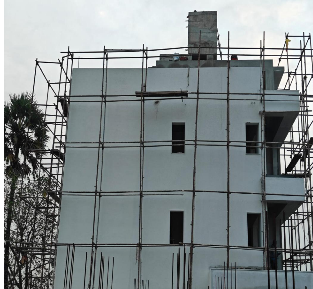
Villa no 16 - External Wall Bubble Texture and Painting work in Progress
