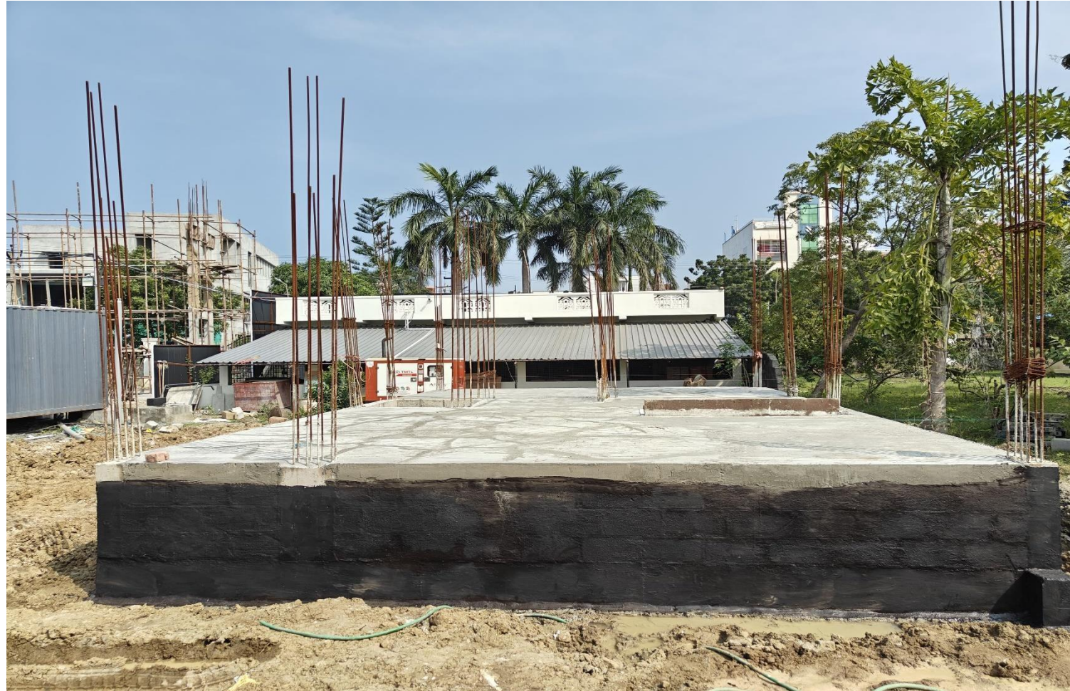
Villa no 03 – Ground Floor Flooring PCC work completed
