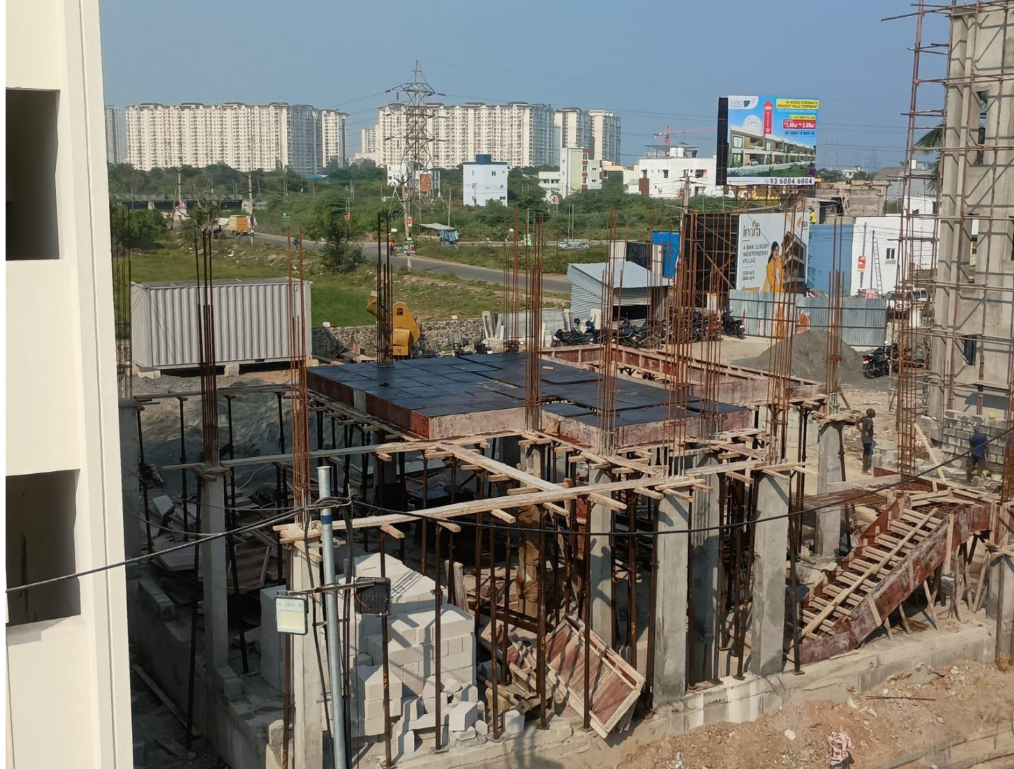
Villa 17 Ground Floor Slab Shuttering work in progress
