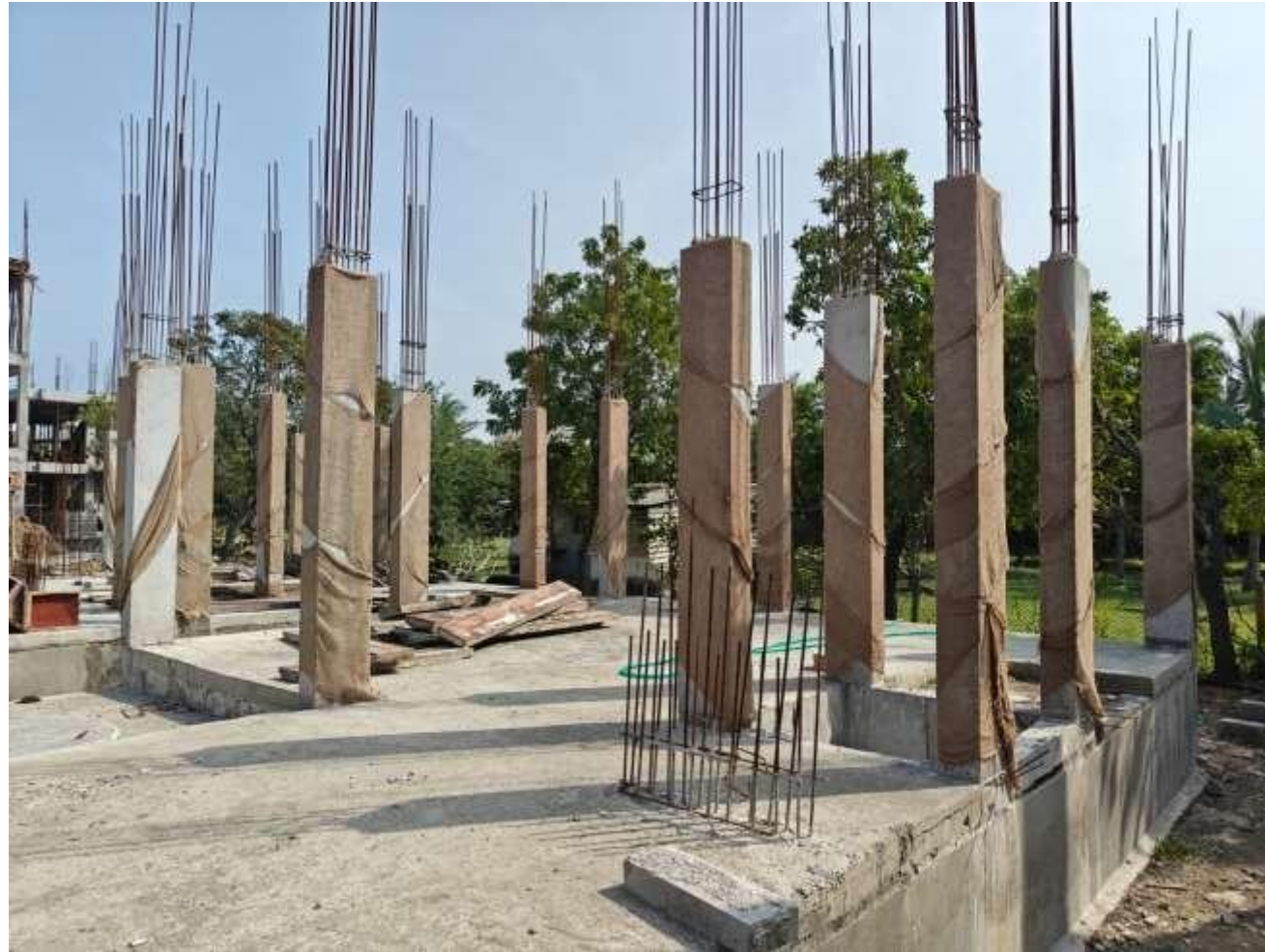
VillaNo 10 – Ground Floor Column Concrete Work completed
