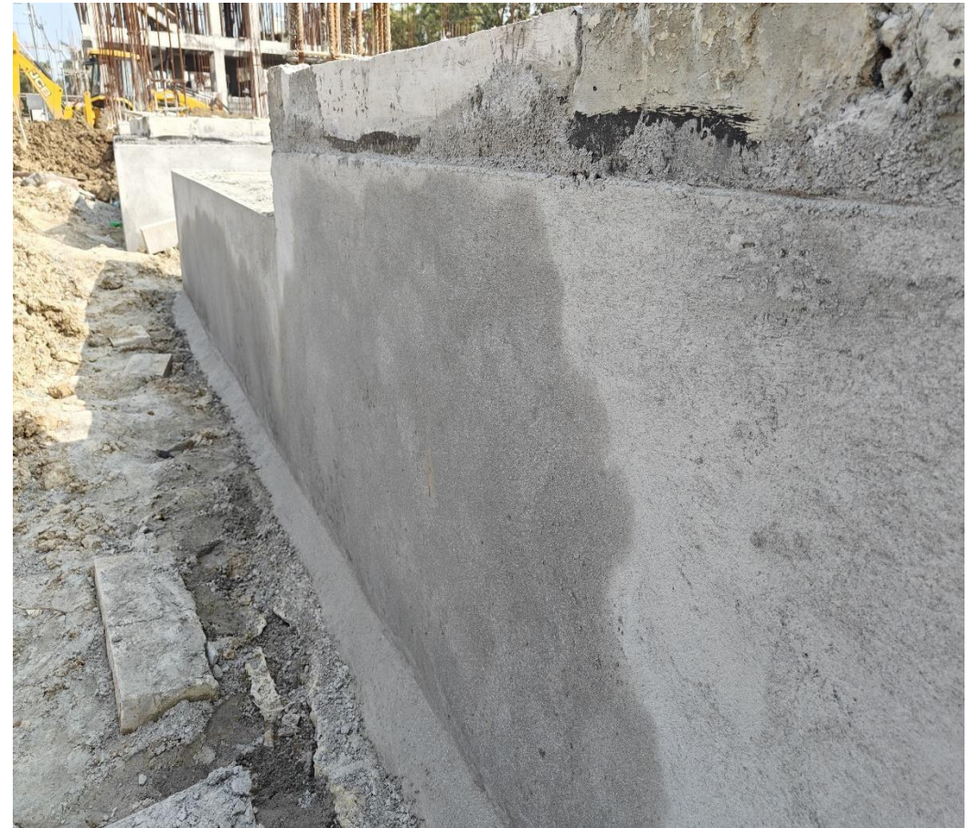
VillaNo 09 , 10 – Basement DPC Protection Plastering work completed
