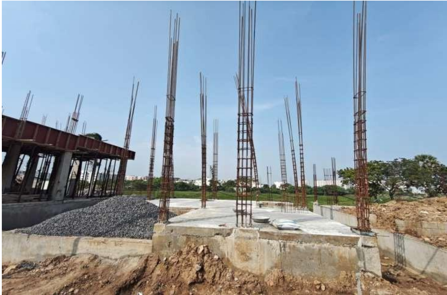
VillaNo 13 – Ground Floor PCC Concrete work completed
