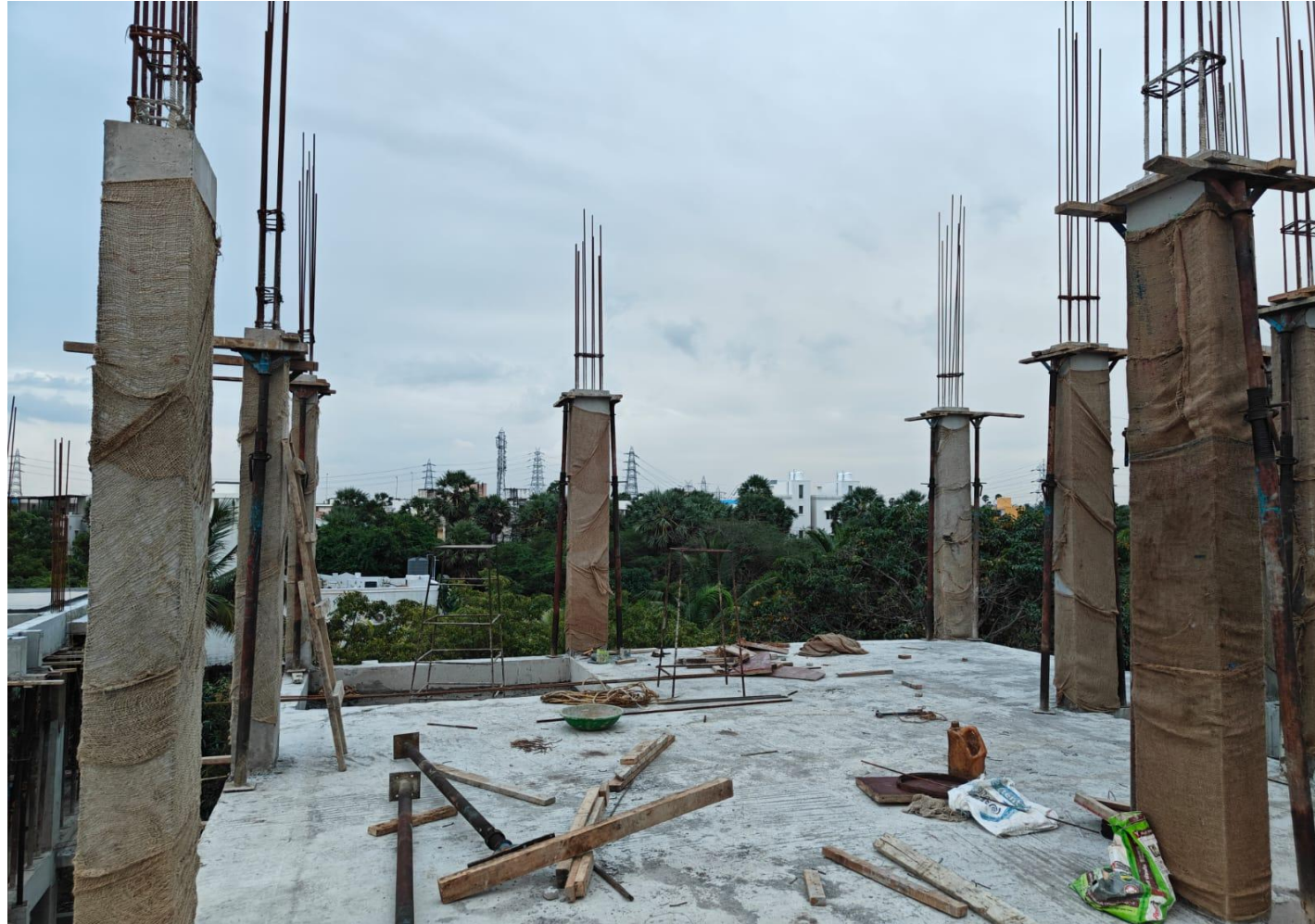
Villa no 06 – Second Floor column concrete work completed
