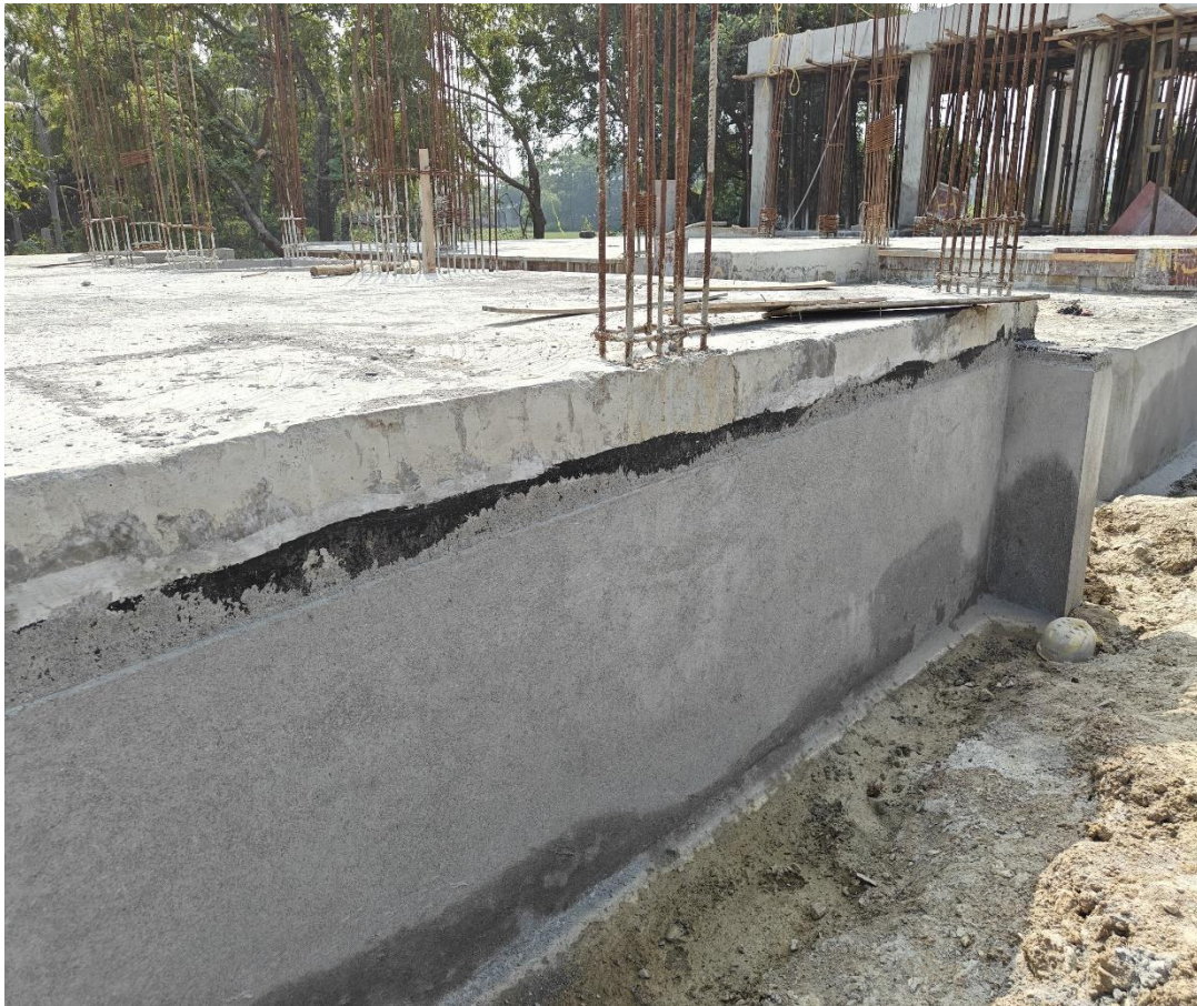
VillaNo 09 , 10 – Basement DPC Protection Plastering work completed
