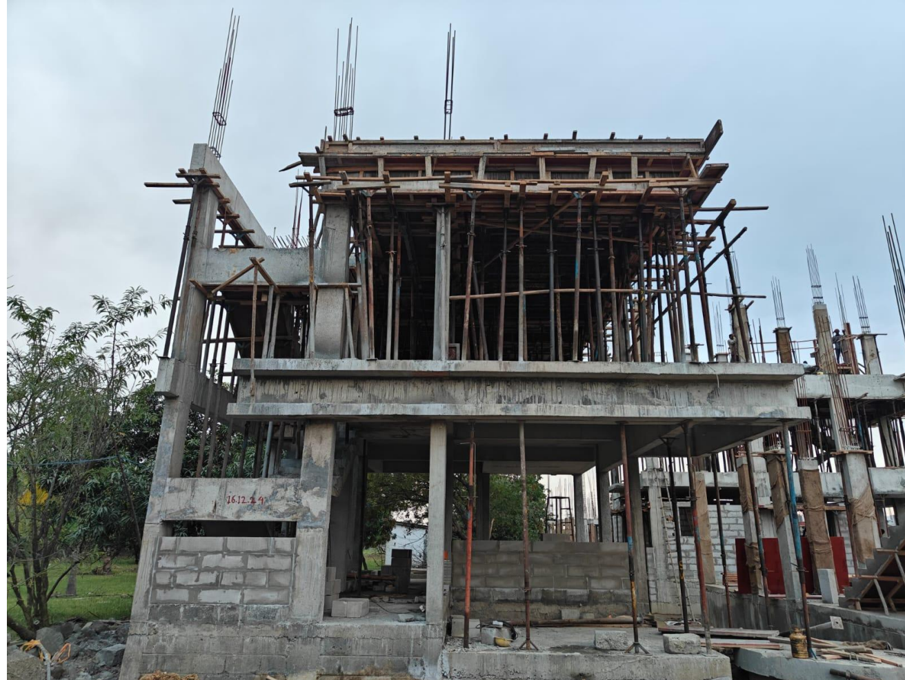
Villa No 4 – First Floor Roof Slab Concrete Completed
