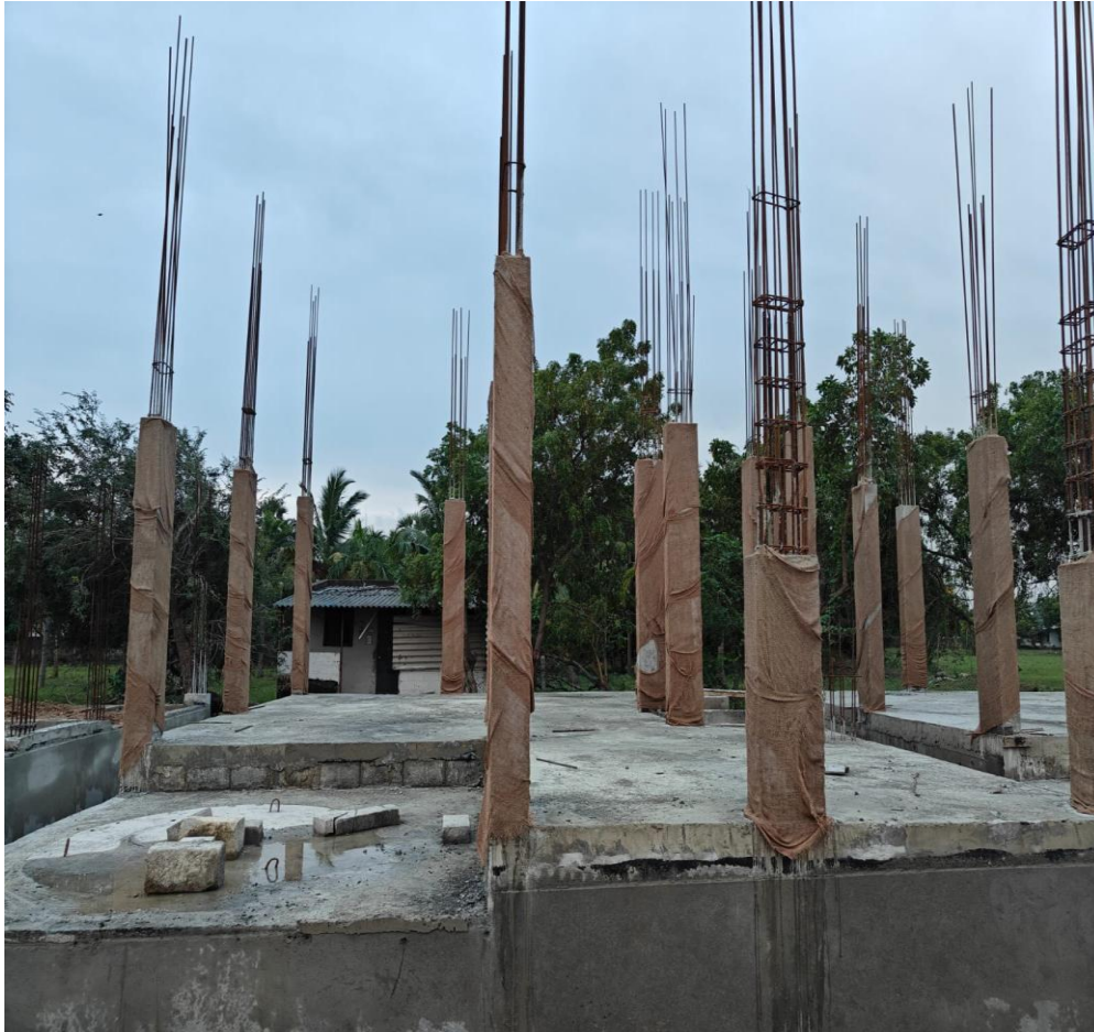
Villa No 09 , 10 – GF Column Concrete Work completed
