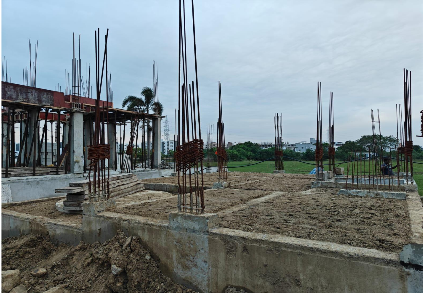
Villa No 13 – Ground Floor PCC laying Preparation work in progress
