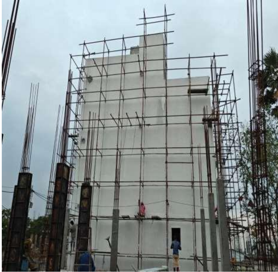
Villa no 16 - External Wall Bubble Texture and Painting work in Progress
