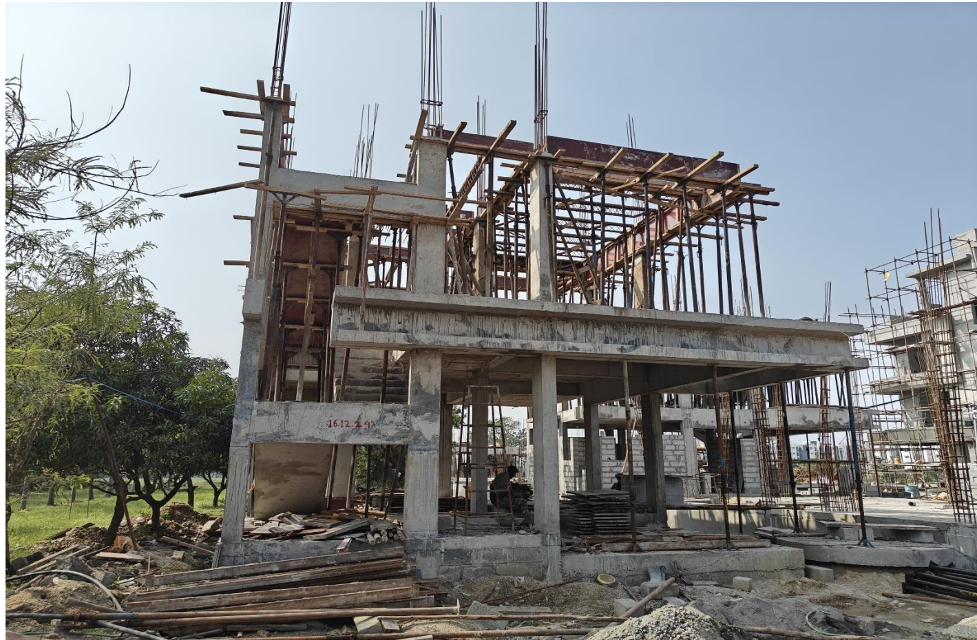
VillaNo 4 – First Floor Roof Slabshuttering work in Progress
