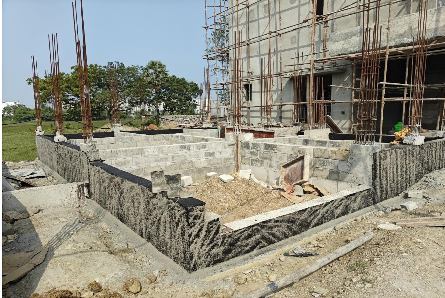
Villa no 14 – Basement DPC coating work in progress
