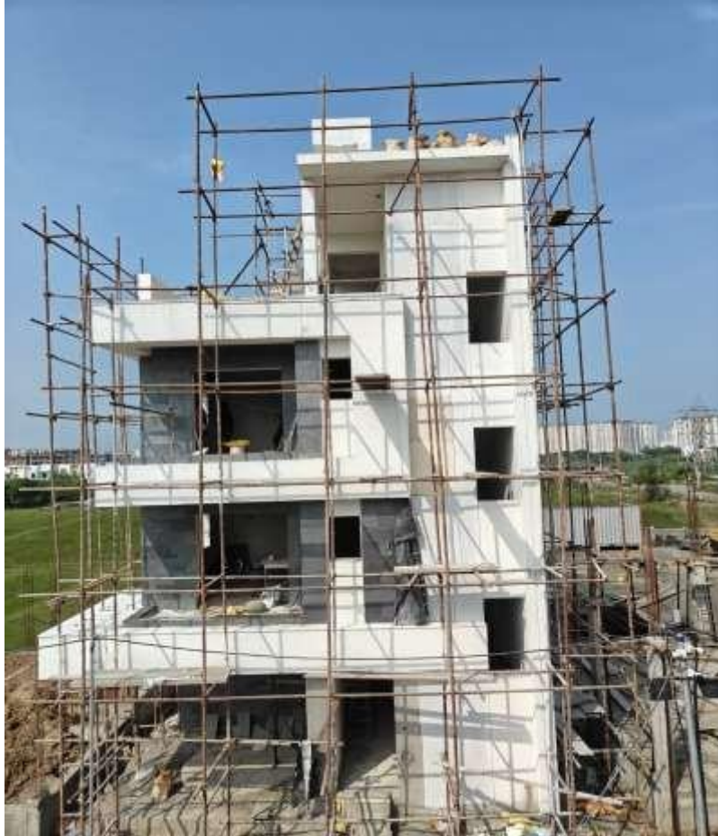
Villa no 16 – External Wall Pebble Texture and Painting work in Progress
