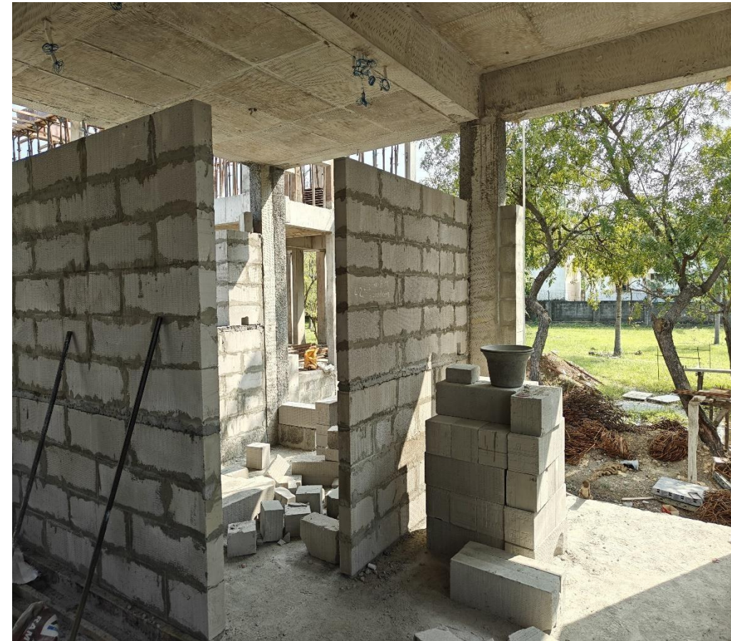
VillaNo 06 – Ground Floor Blockwork in progress
