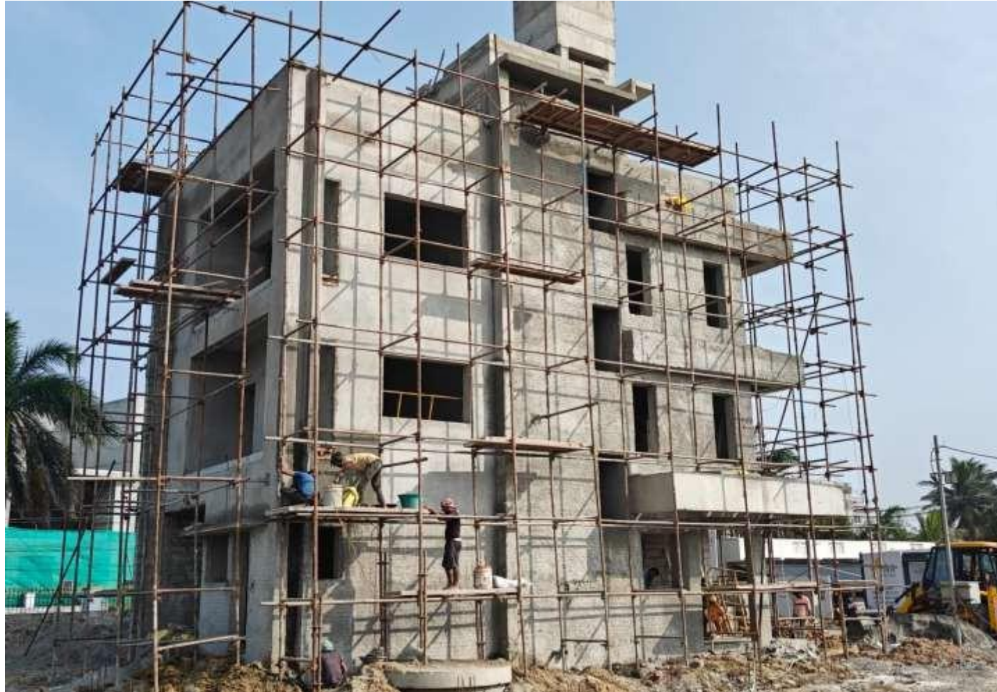
VillaNo 20– External wall plastering work in progress
