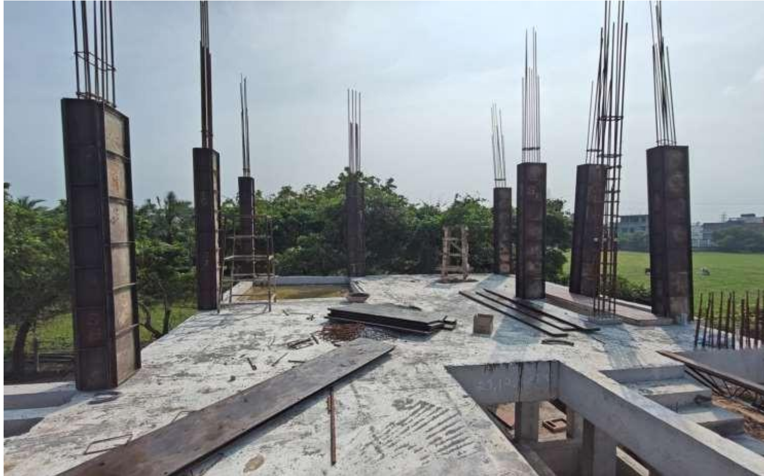
VillaNo 11 – First Floor Column Shuttering Work in progress
