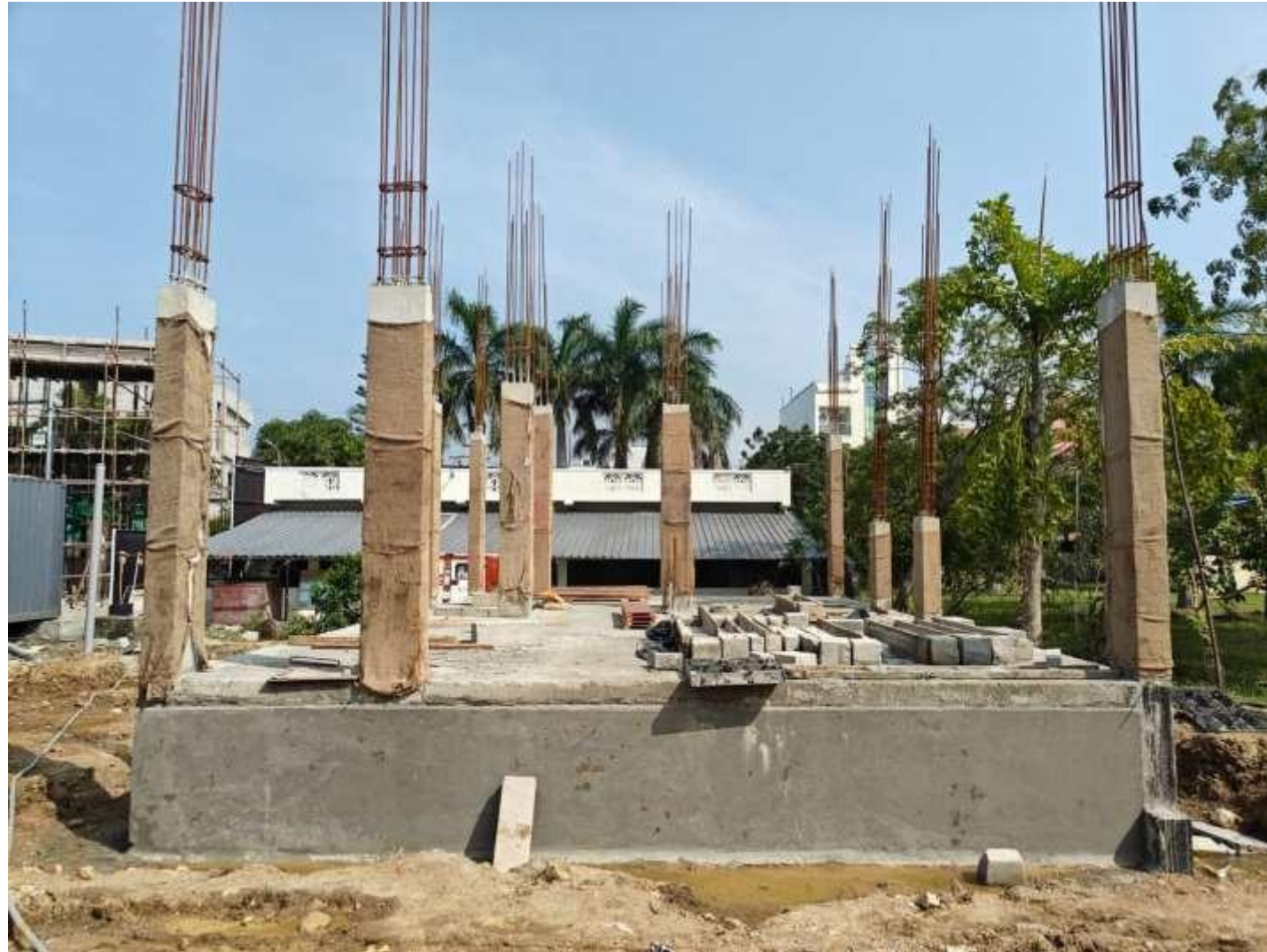
Villa no 03 – Ground Floor Column Concrete work completed
