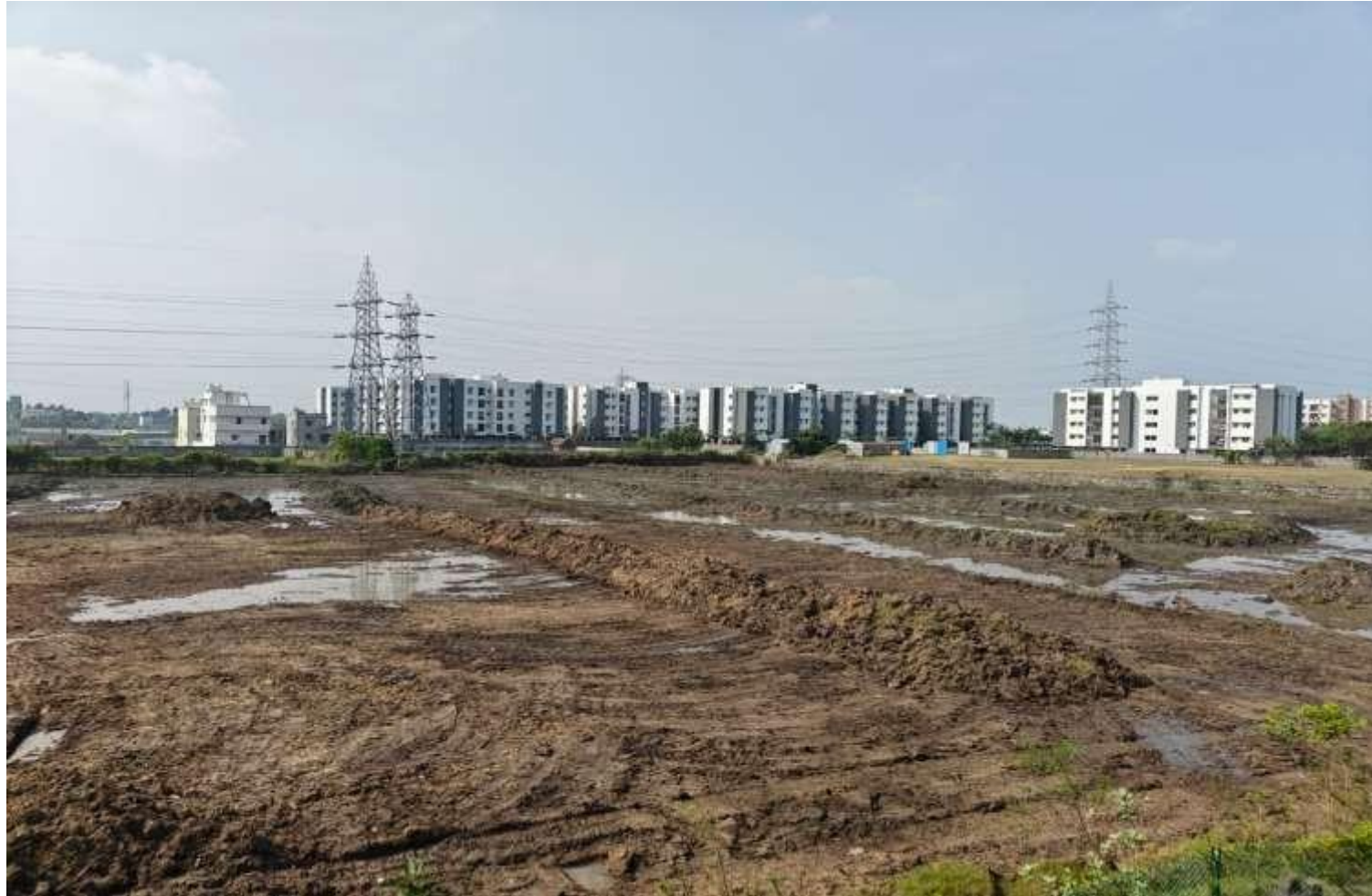
Phase 2 - Boundary bushes Cleaning work in progress
