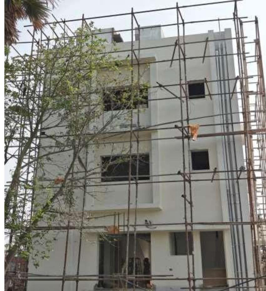
Villa no 16 – External Wall Pebble Texture and Painting work in Progress
