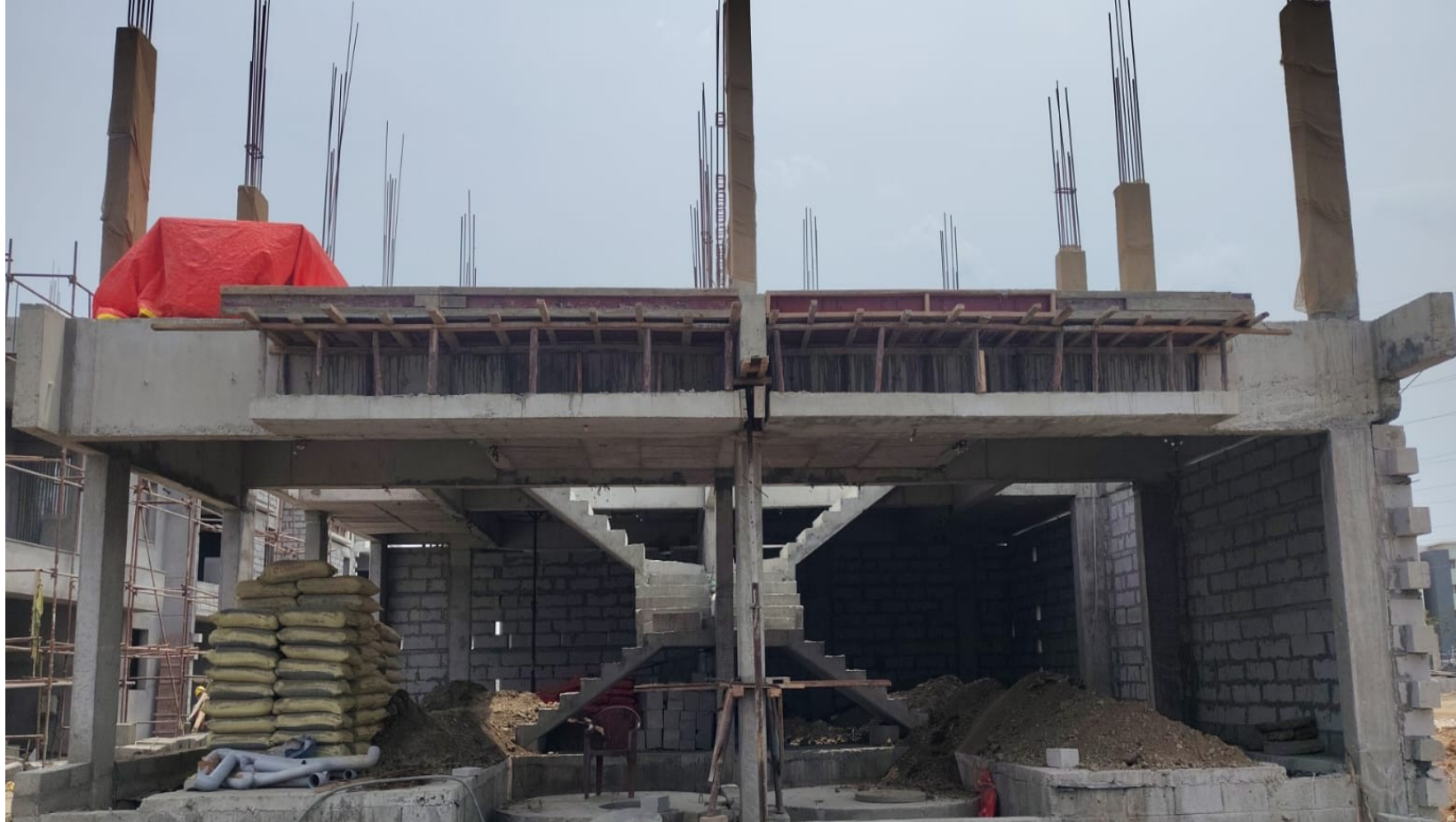
Villa No 97 to 98 –FF Column Concrete Pouring Completed
