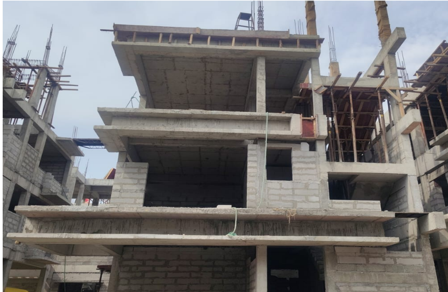
Villa No 42 – FF Block Work In Progress
