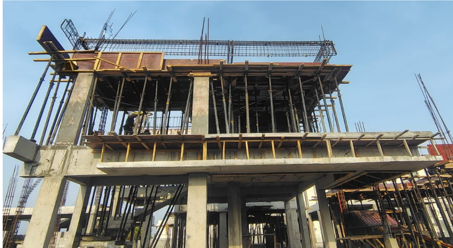
Villa No 114-FF Roof Slab Reinforcement Work In Progress
