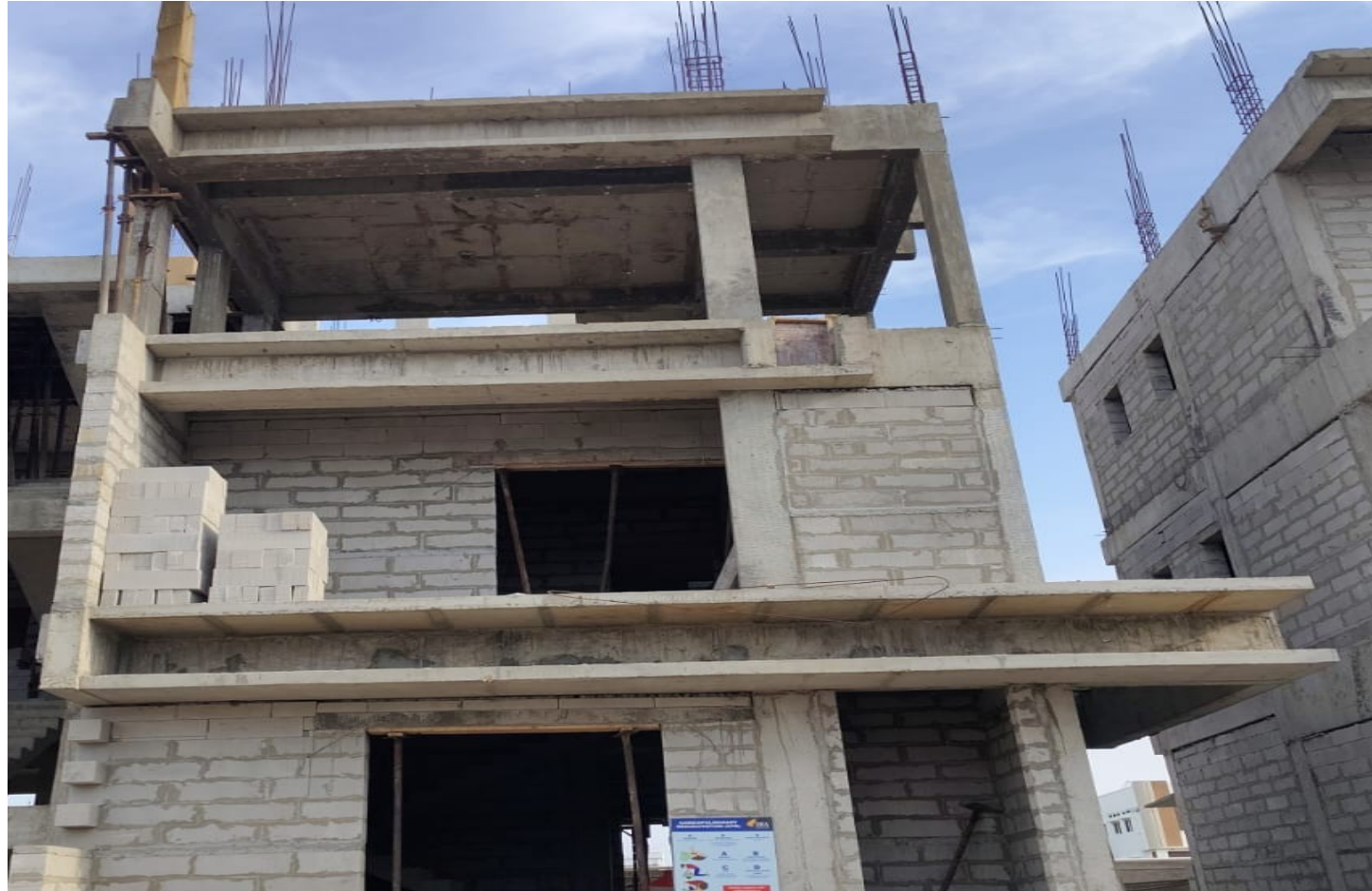
Villa No 28 –Head Room Roof Slab Column Concrete Pouring Completed
