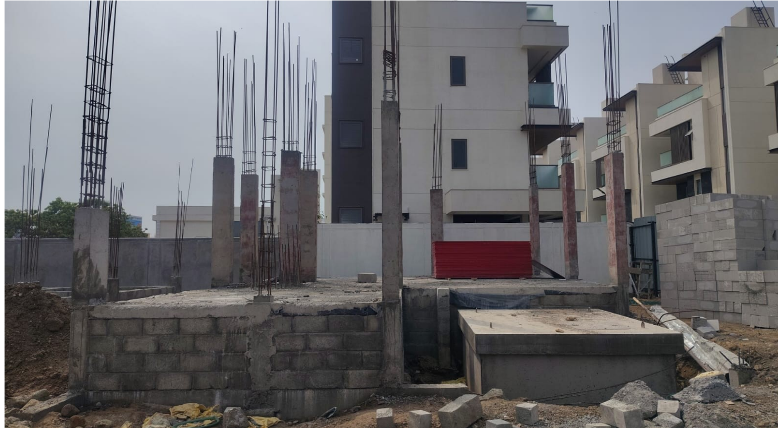
Villa No 123–GF Colum Concrete Pouring Work Completed
