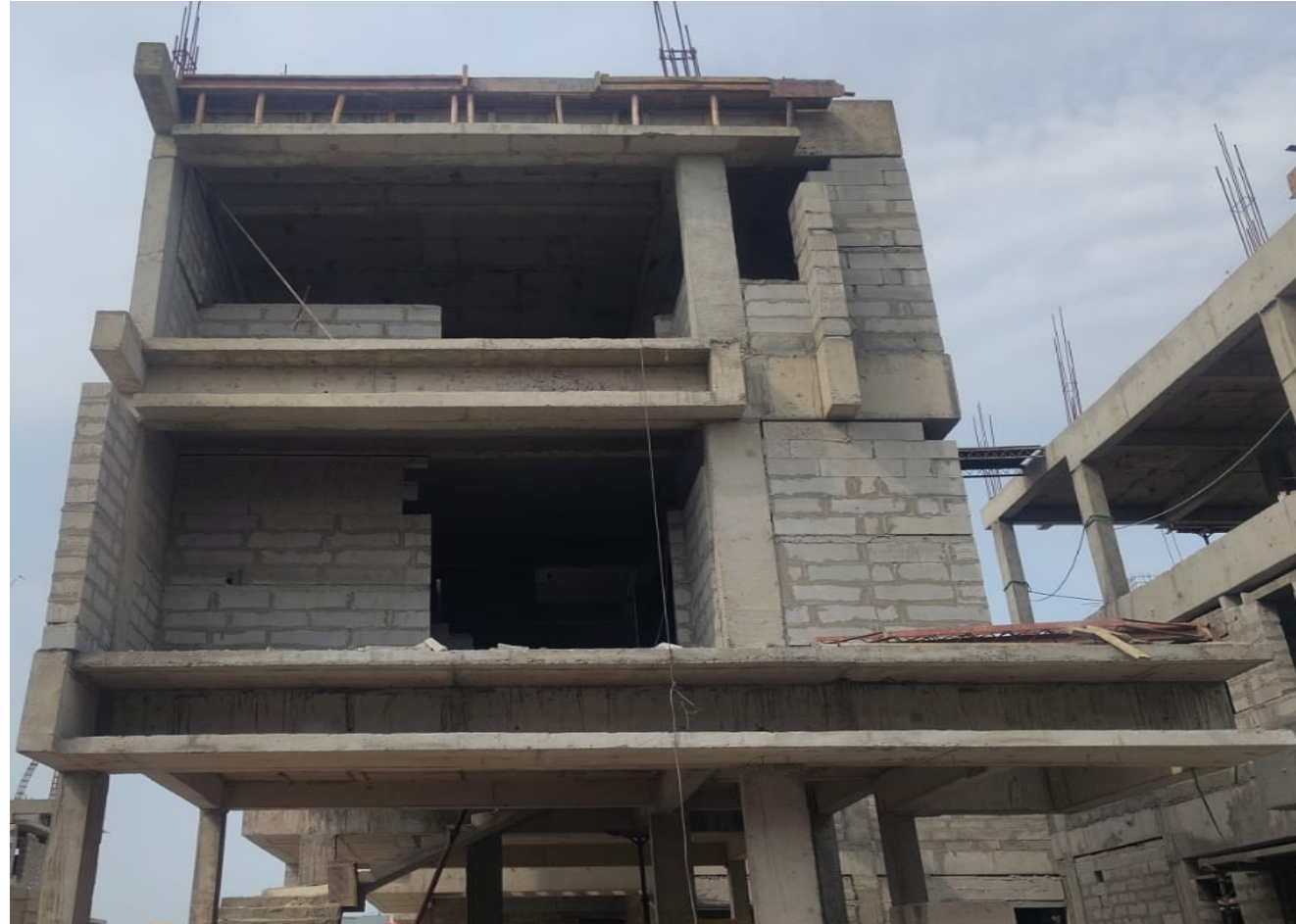
Villa No 41- SF Block work In Progress
