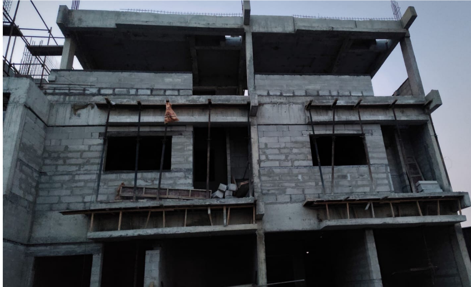
Villa No 101 to 102– FF Block Work In Progress
