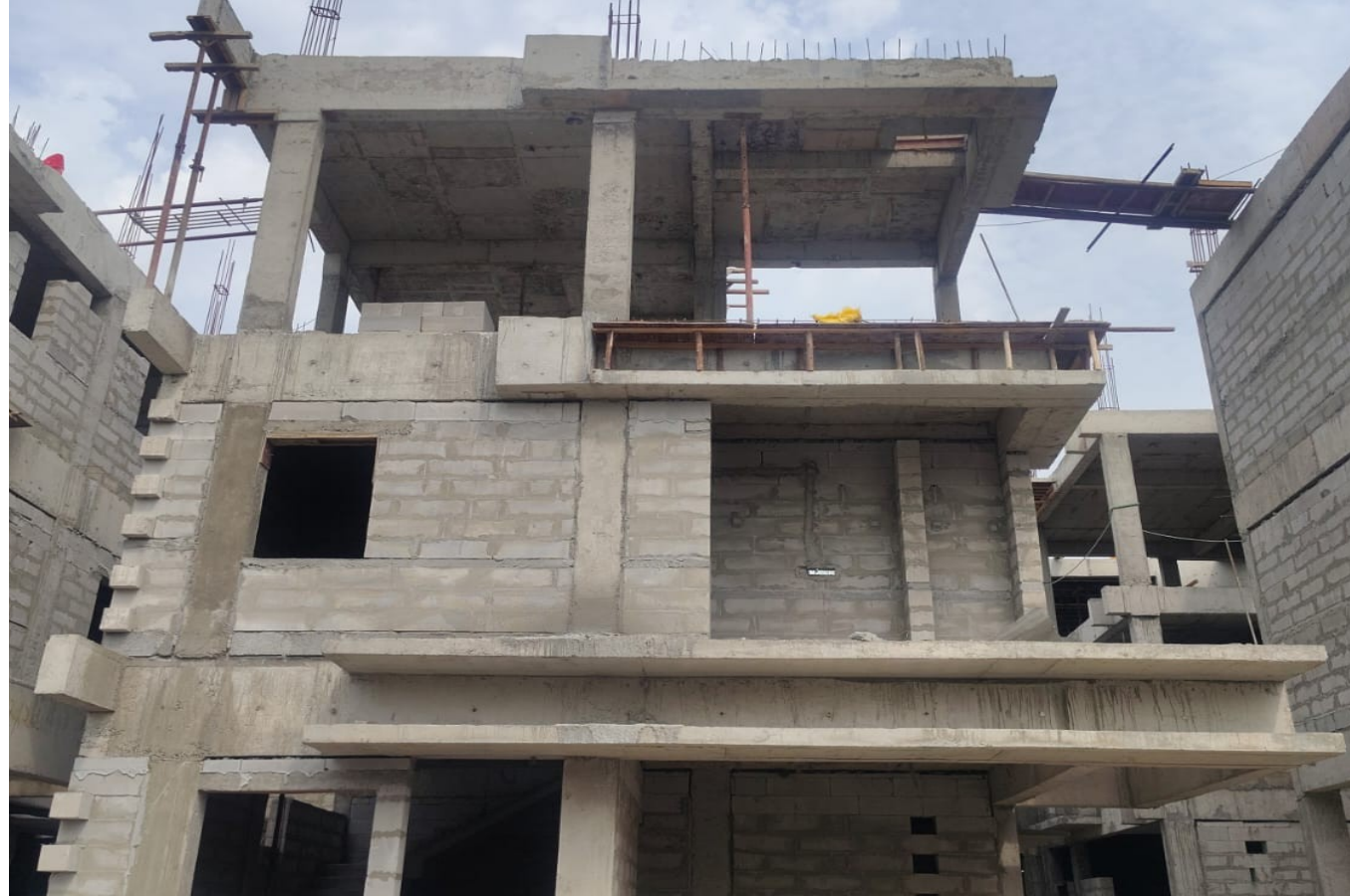
Villa No 40–SF Block Work In Progress
