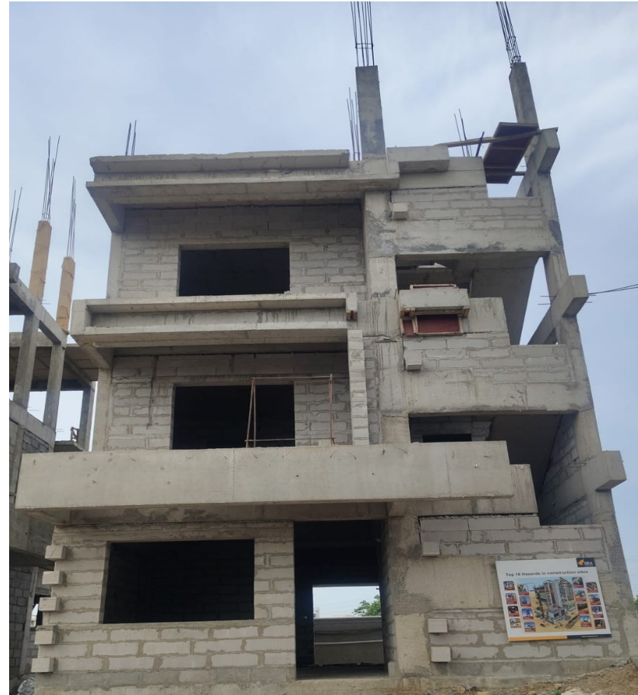
Villa No-29 Head Room Column Concrete work Completed
