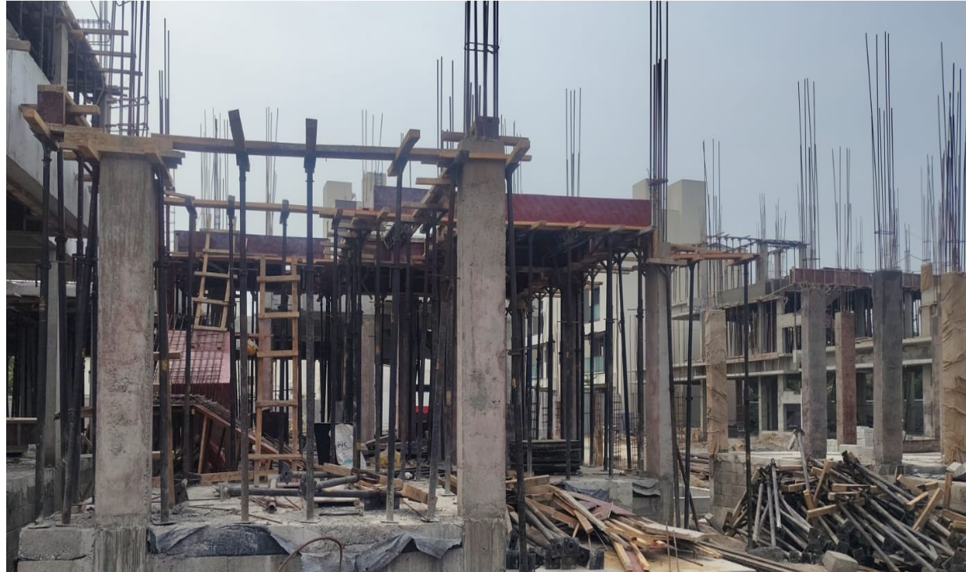
Villa No 115–GF Roof Slab Shuttering Work In Progress
