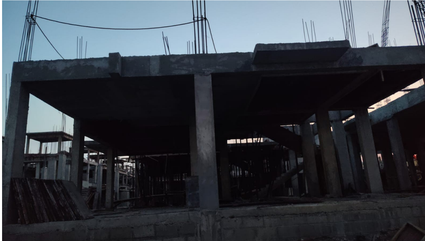
Villa No 103–GF Roof Slab Concrete Pouring Work Completed
