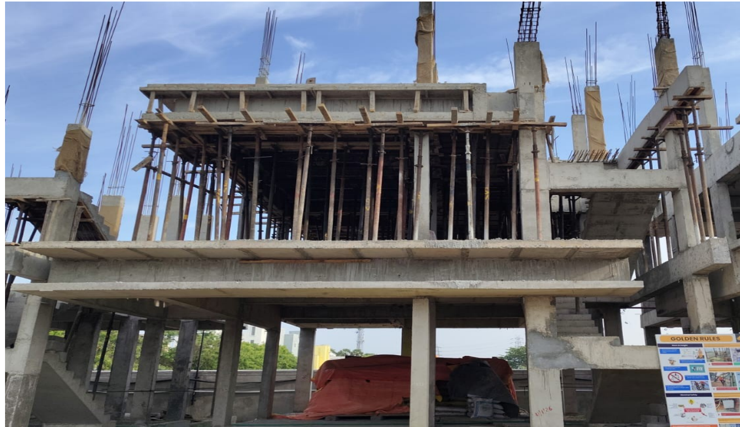
Villa No 25- SF Column Concrete Pouring Completed
