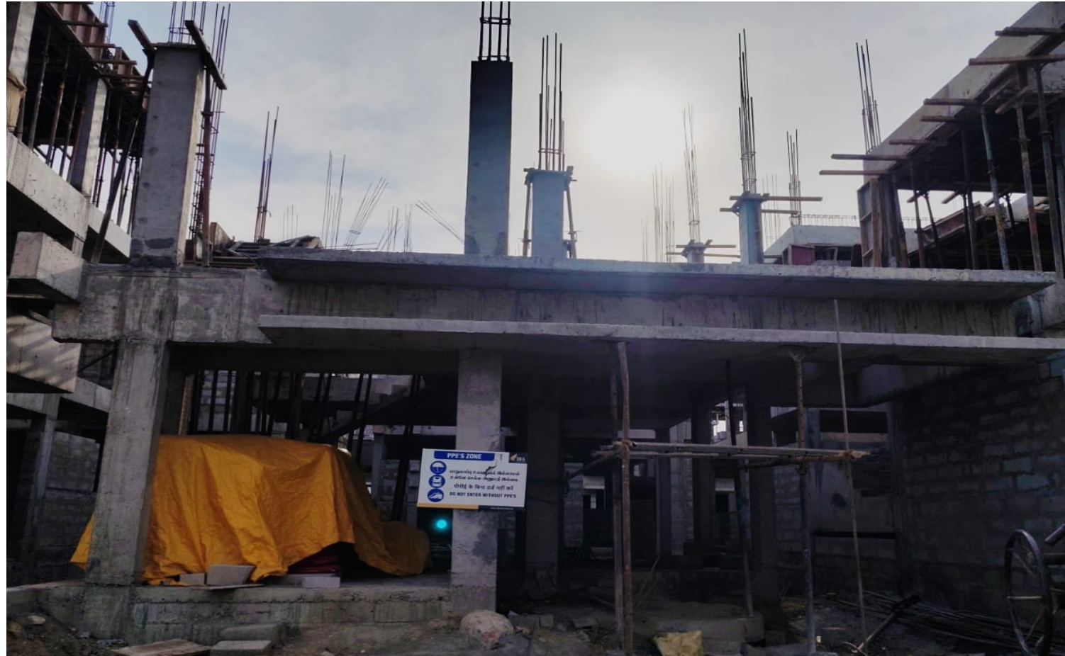
Villa No 31- FF Column Concrete Pouring Completed
