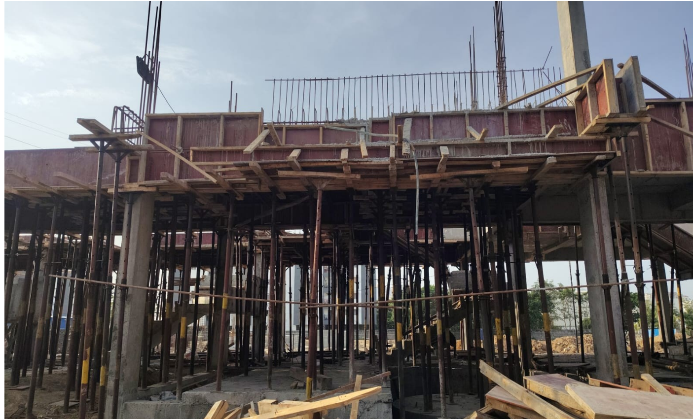
Villa No 90 –FF Column Concrete Pouring Work Completed
