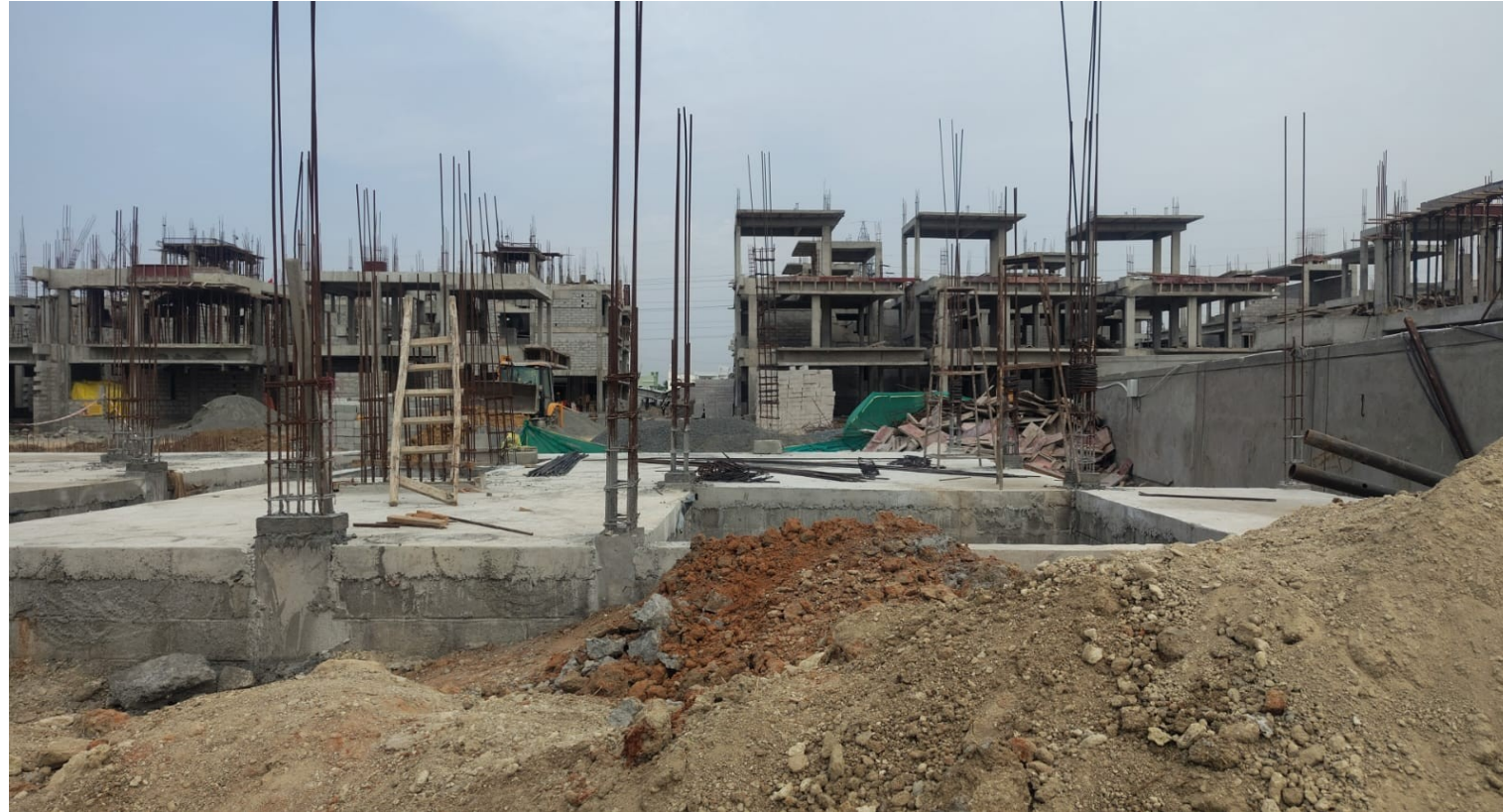
Villa No 112–GF Column Starter Concrete Completed
