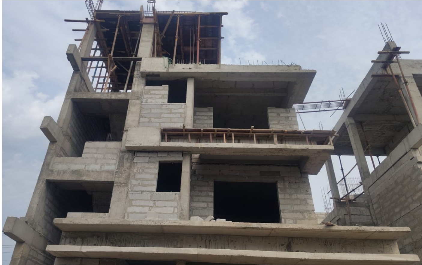
Villa No 39 –Head Room Slab Reinforcement Work In Progress
