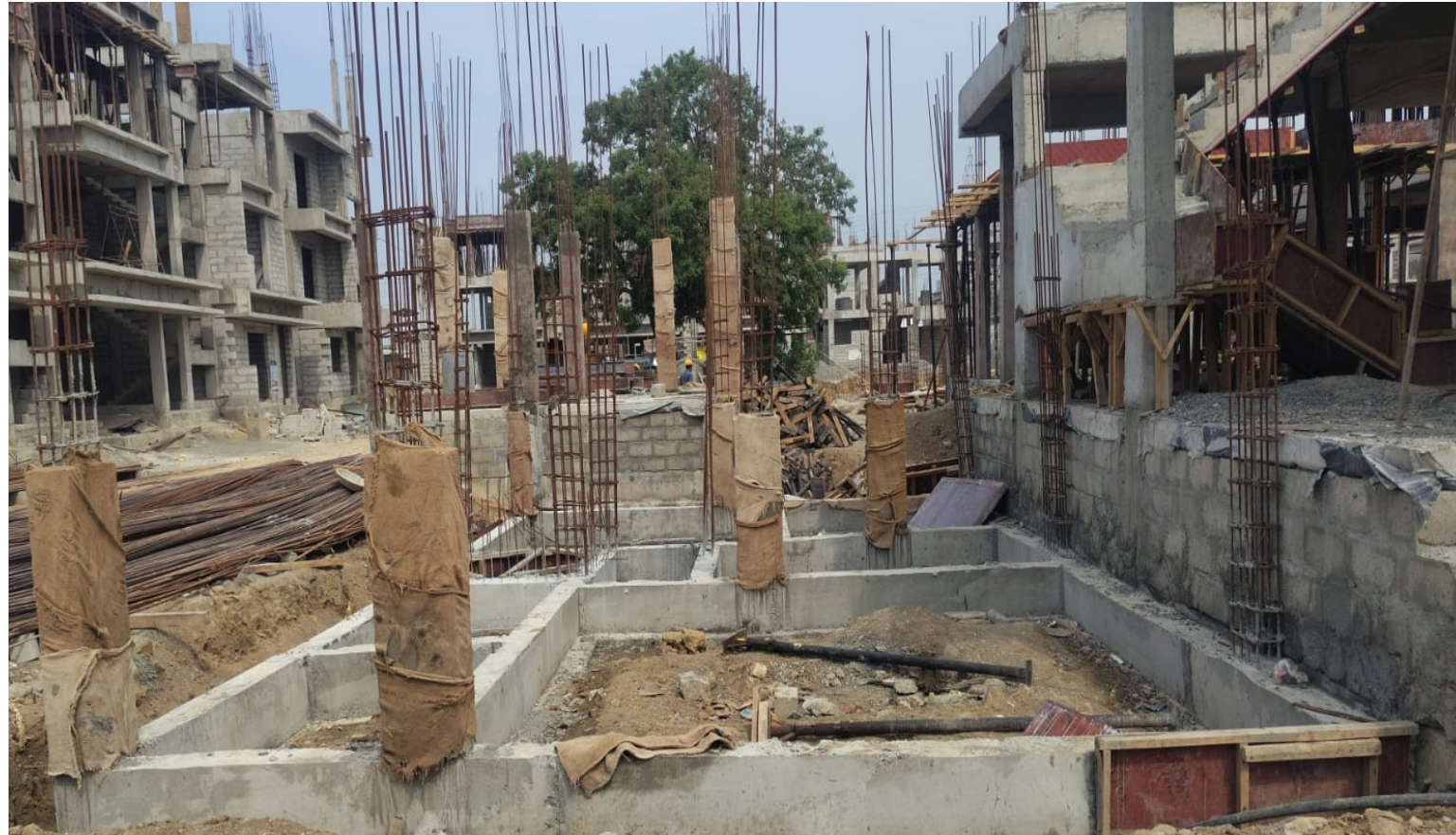
Villa No 117–Basement Column Concrete Pouring Completed
