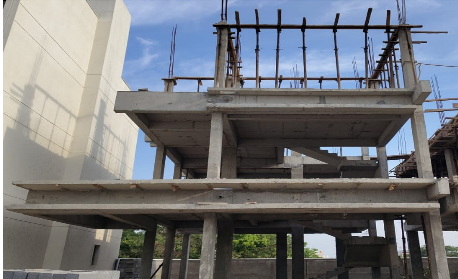
Villa No 22 –SF Roof Slab Shuttering work In Progress
