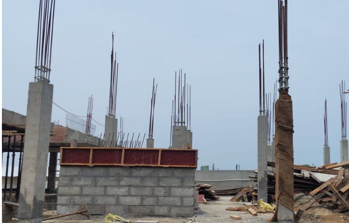
Villa No 107–GF Column Concrete Pouring Completed
