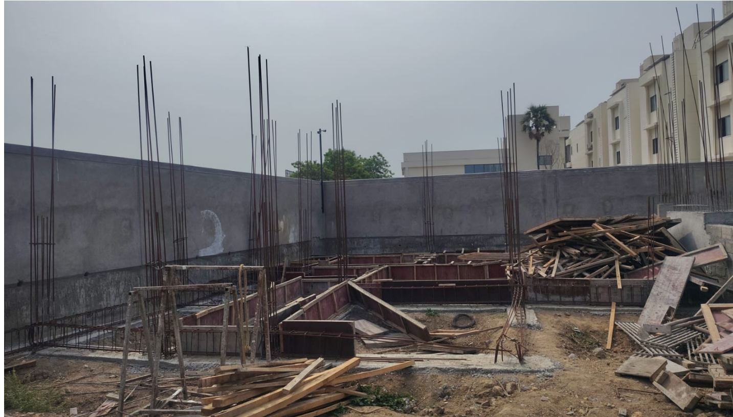
Villa No 121–Plinth Beam Shuttering Work In Progress
