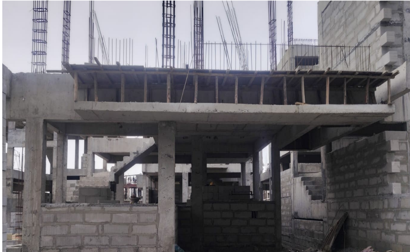
Villa No 36–FF Column Reinforcement Work In Progress
