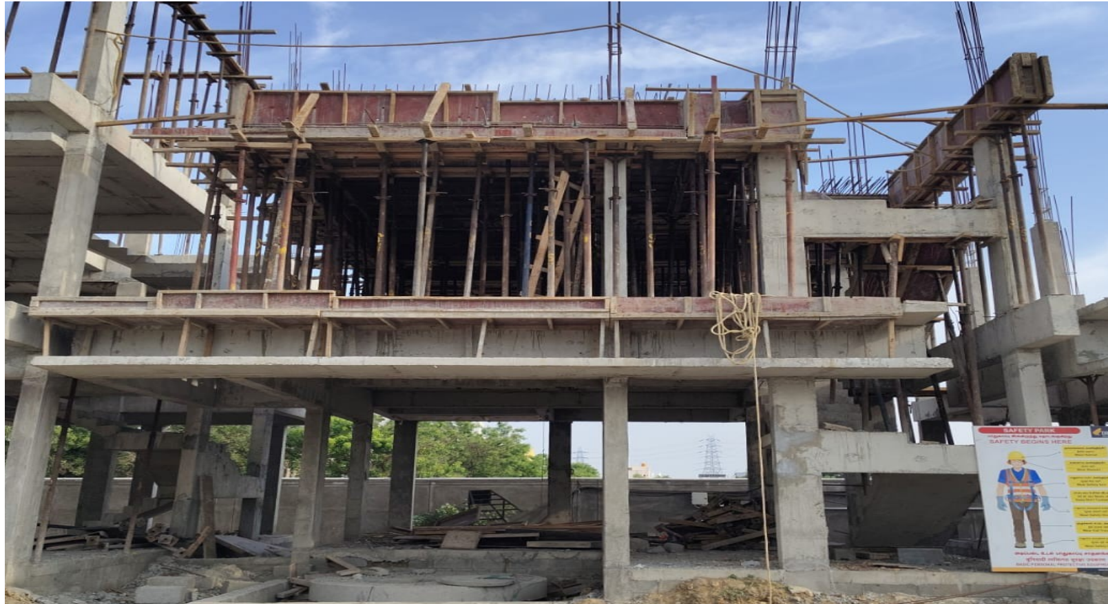
Villa No 23 –FF Roof Slab Concrete Pouring Work Completed
