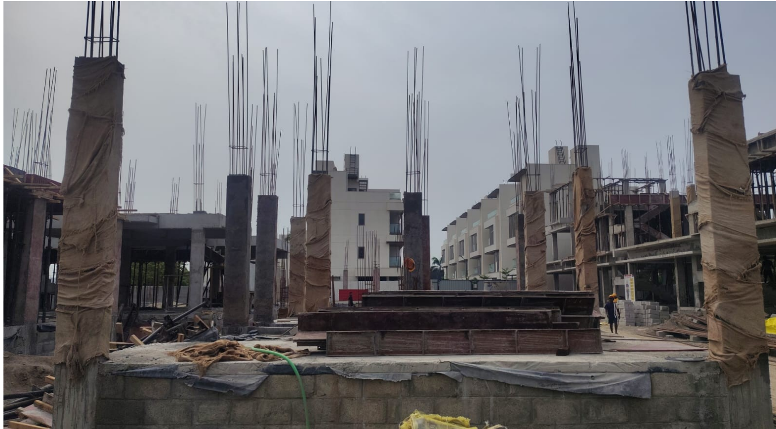
Villa No 116–GF Column Concrete Pouring Work Completed
