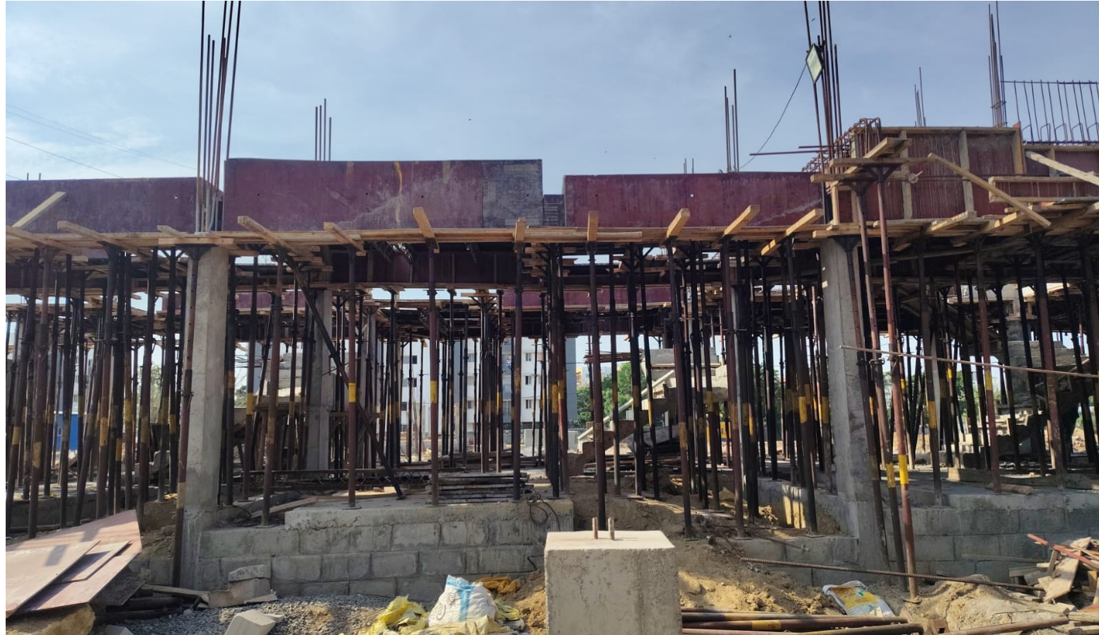
Villa No 87 To 89 –GF Roof Slab Shuttering Work In Progress
