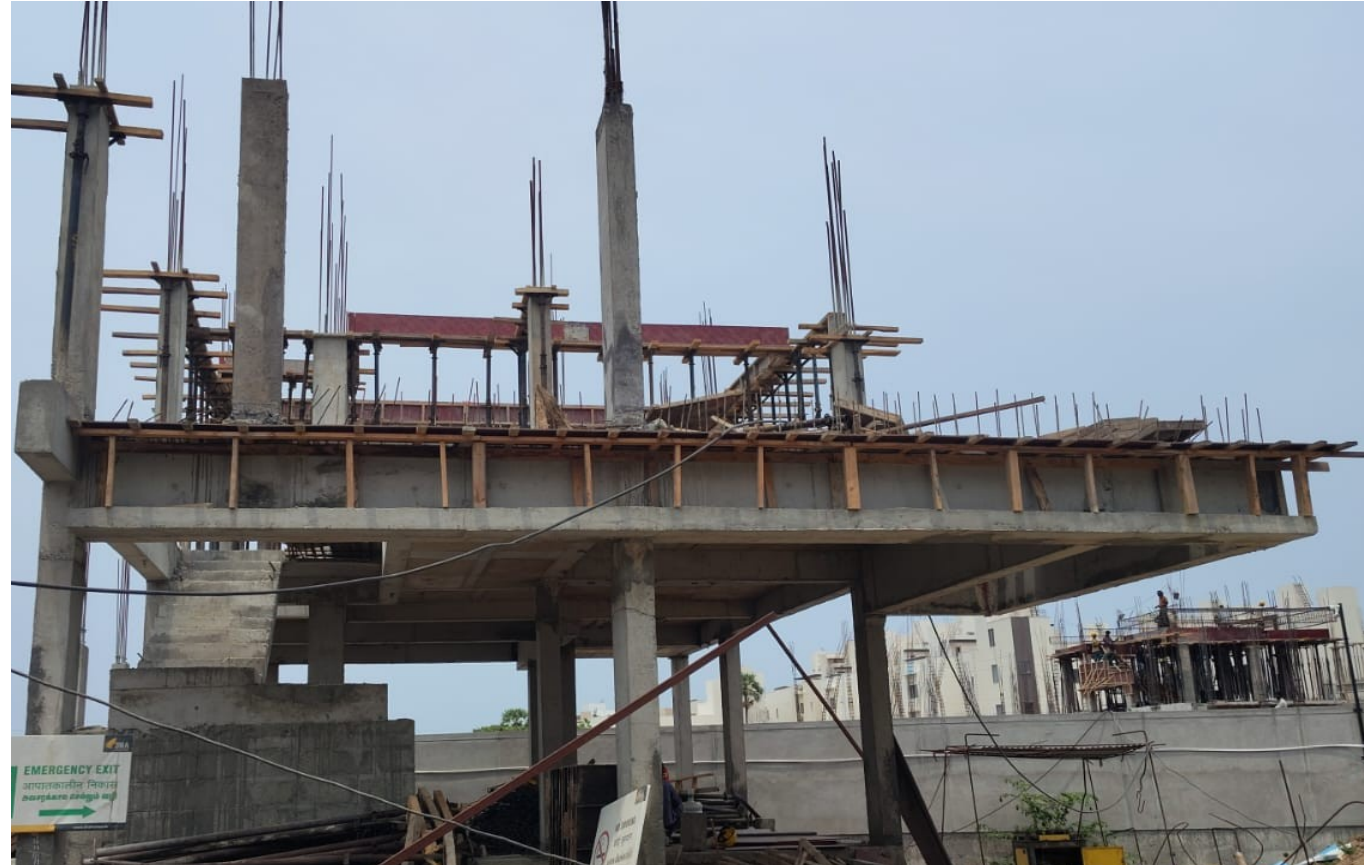
Villa No 108–FF Roof Slab Shuttering work In Progress
