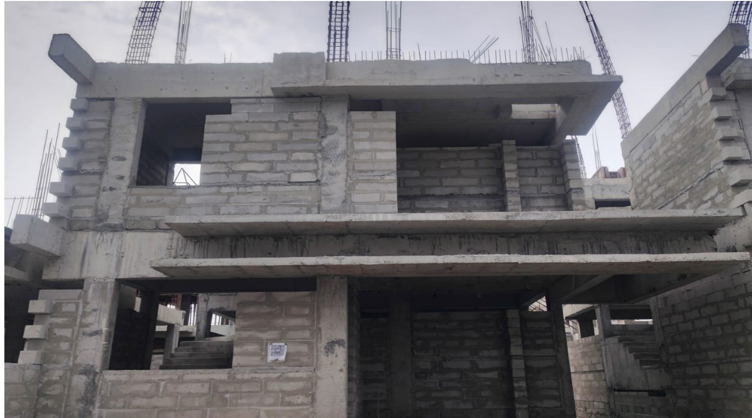
Villa No 37 –FF Block Work In Progress
