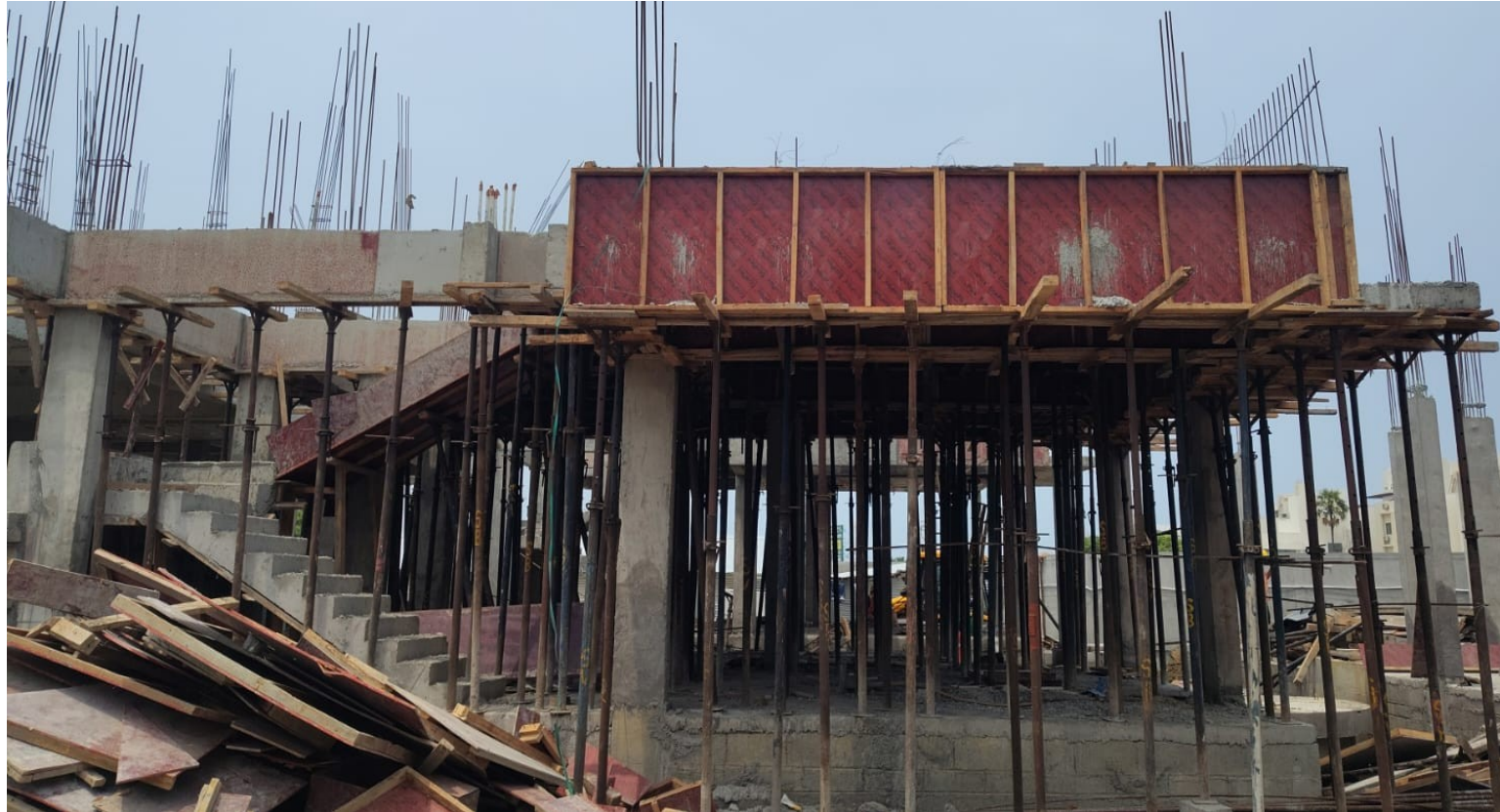
Villa No 106–GF Roof Slab Concrete Pouring Work Completed
