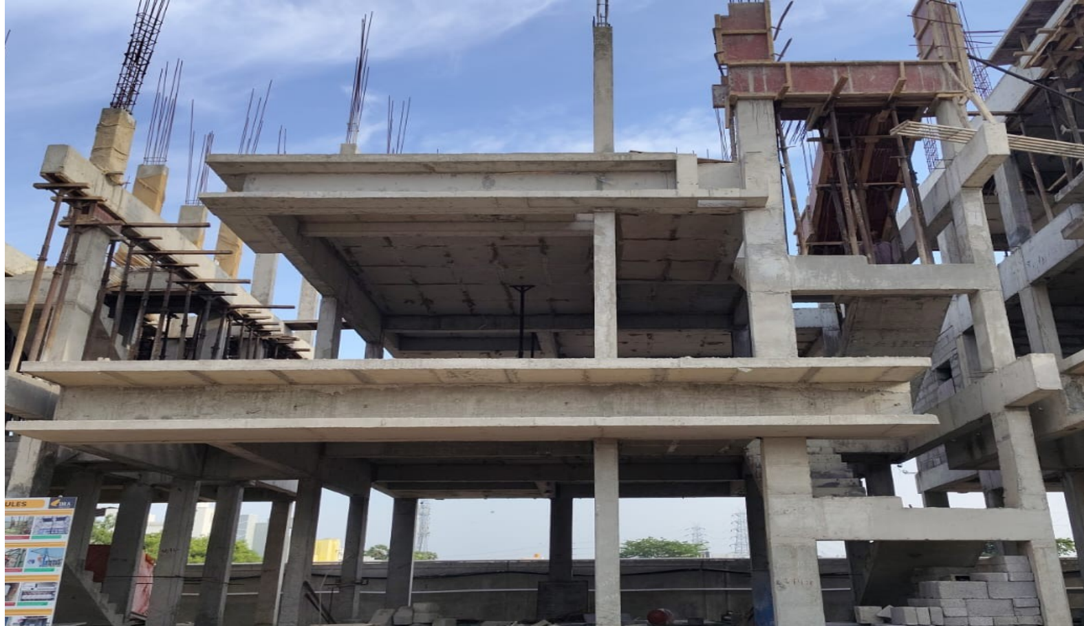
Villa No 26- SF Column Concrete Pouring Completed
