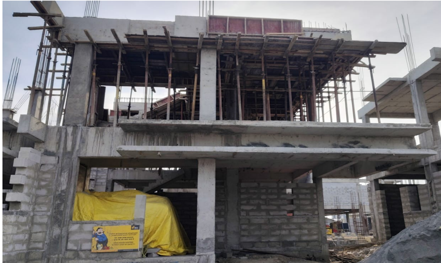
Villa No 32 –FF Roof Slab Concrete Pouring Completed`
