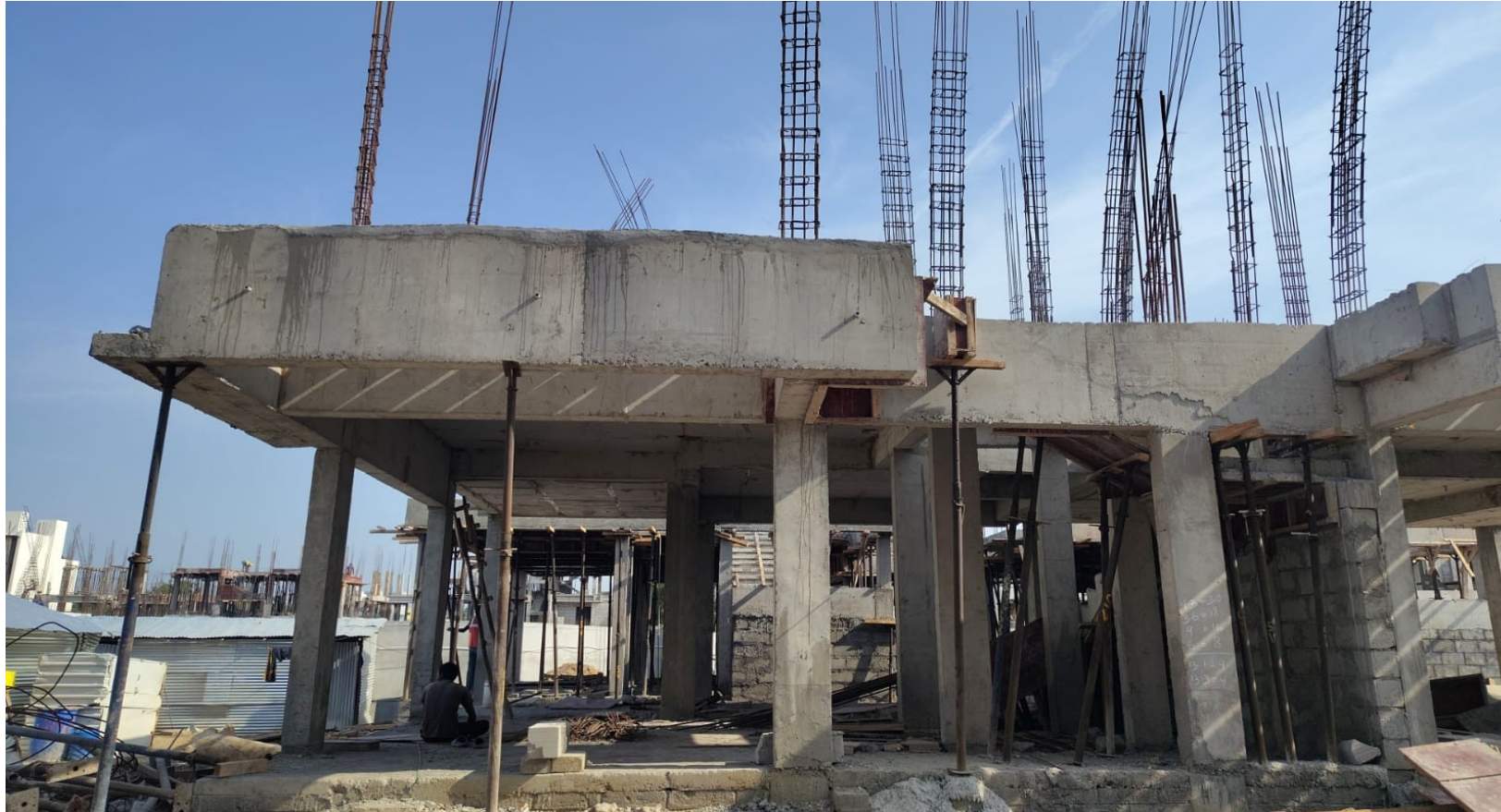
Villa No 104–FF Column Reinforcement Work Completed
