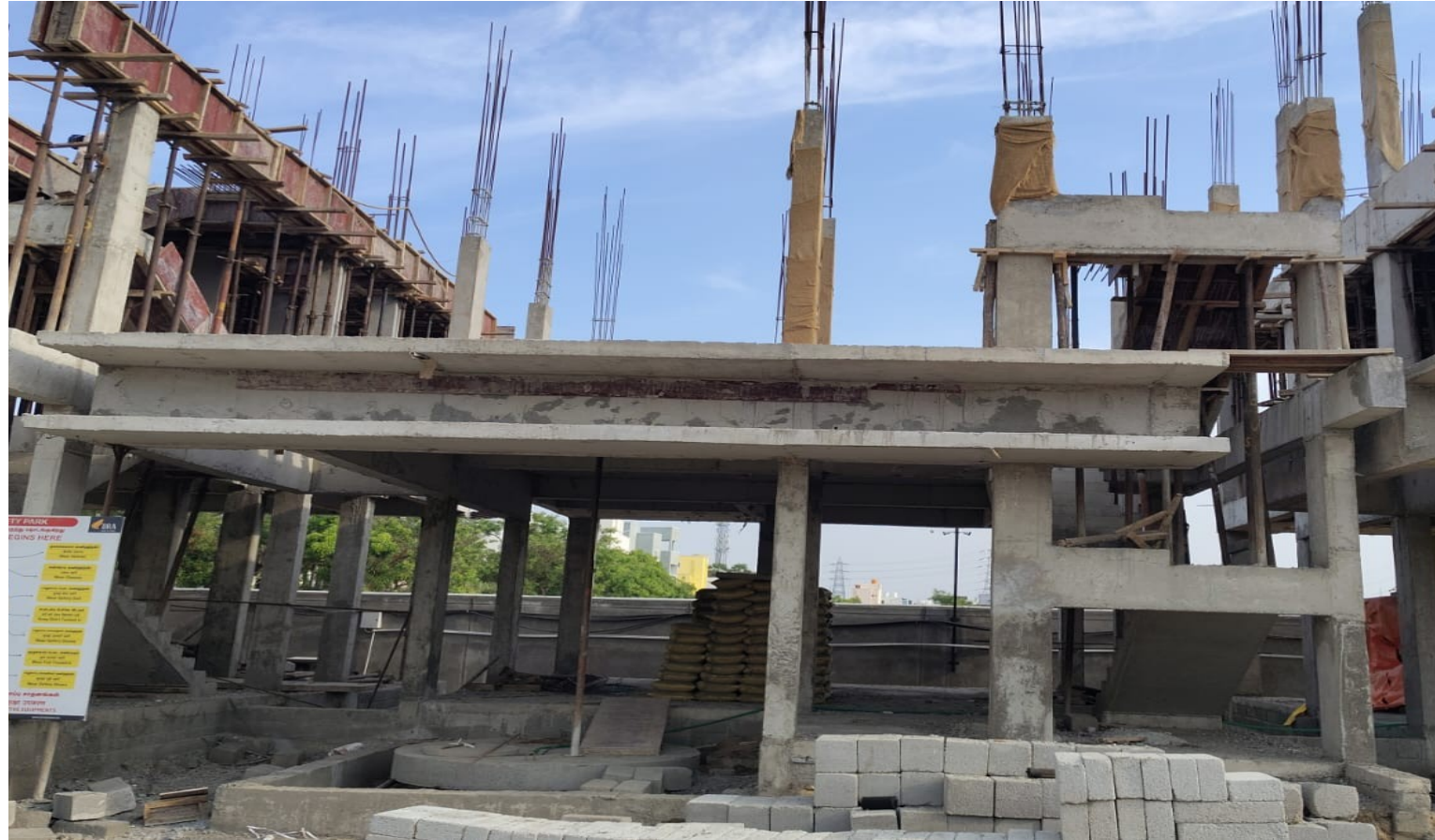
Villa No 24- FF Staircase Mid landing Concrete Completed
