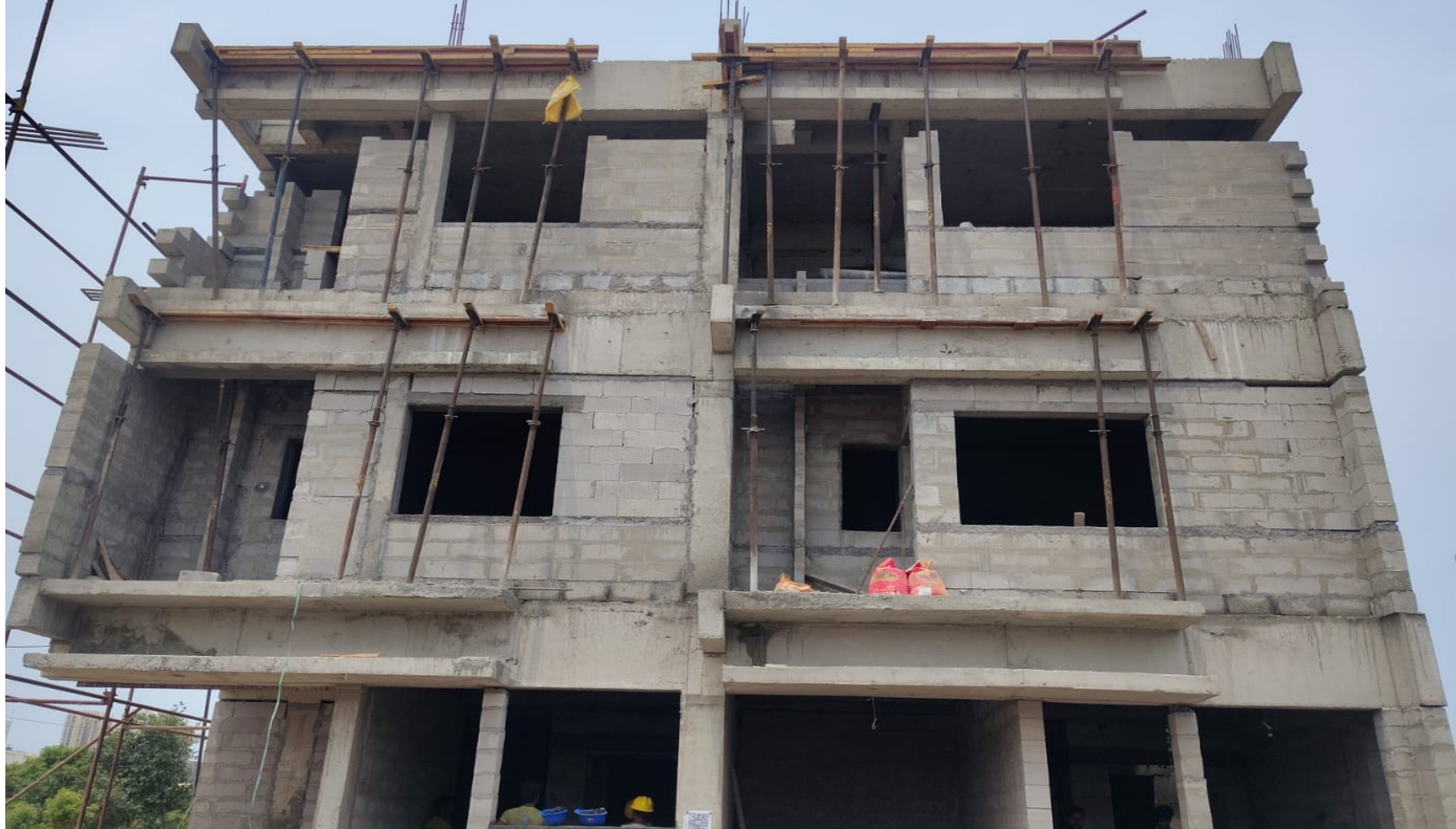
Villa No 99 to 100–SF Block Work In Progress
