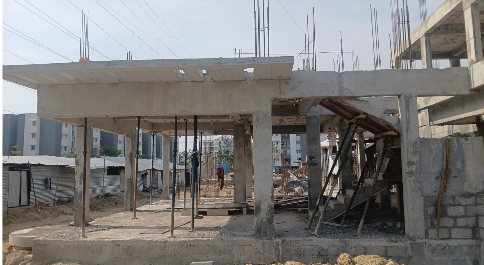
Villa No 62-GF Roof Slab Concrete Pouring Completed
