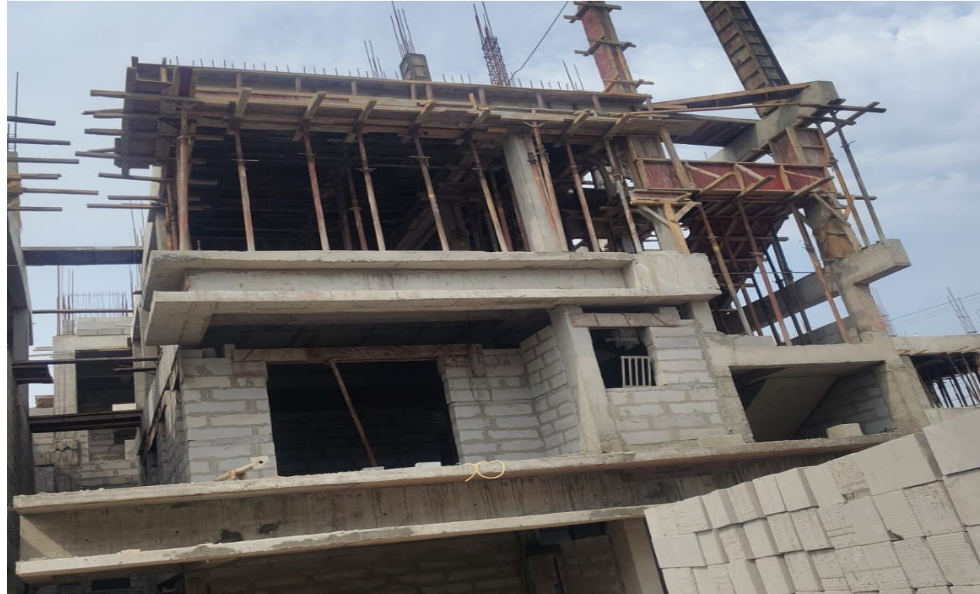
Villa No 43- SF Column Concrete Pouring Work Completed
