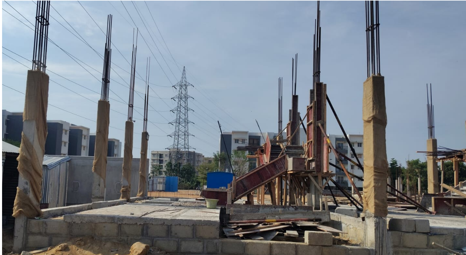
Villa No 83 to 86 –GF Staircase Shuttering Work In Progress
