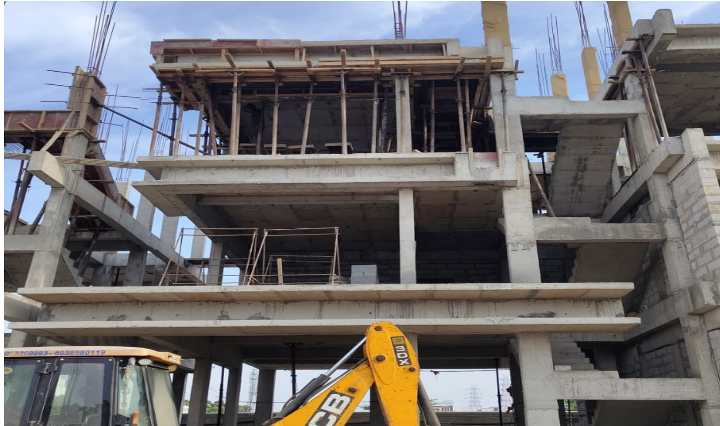
Villa No 27 –Head Room Roof Slab Column Concrete Pouring Completed
