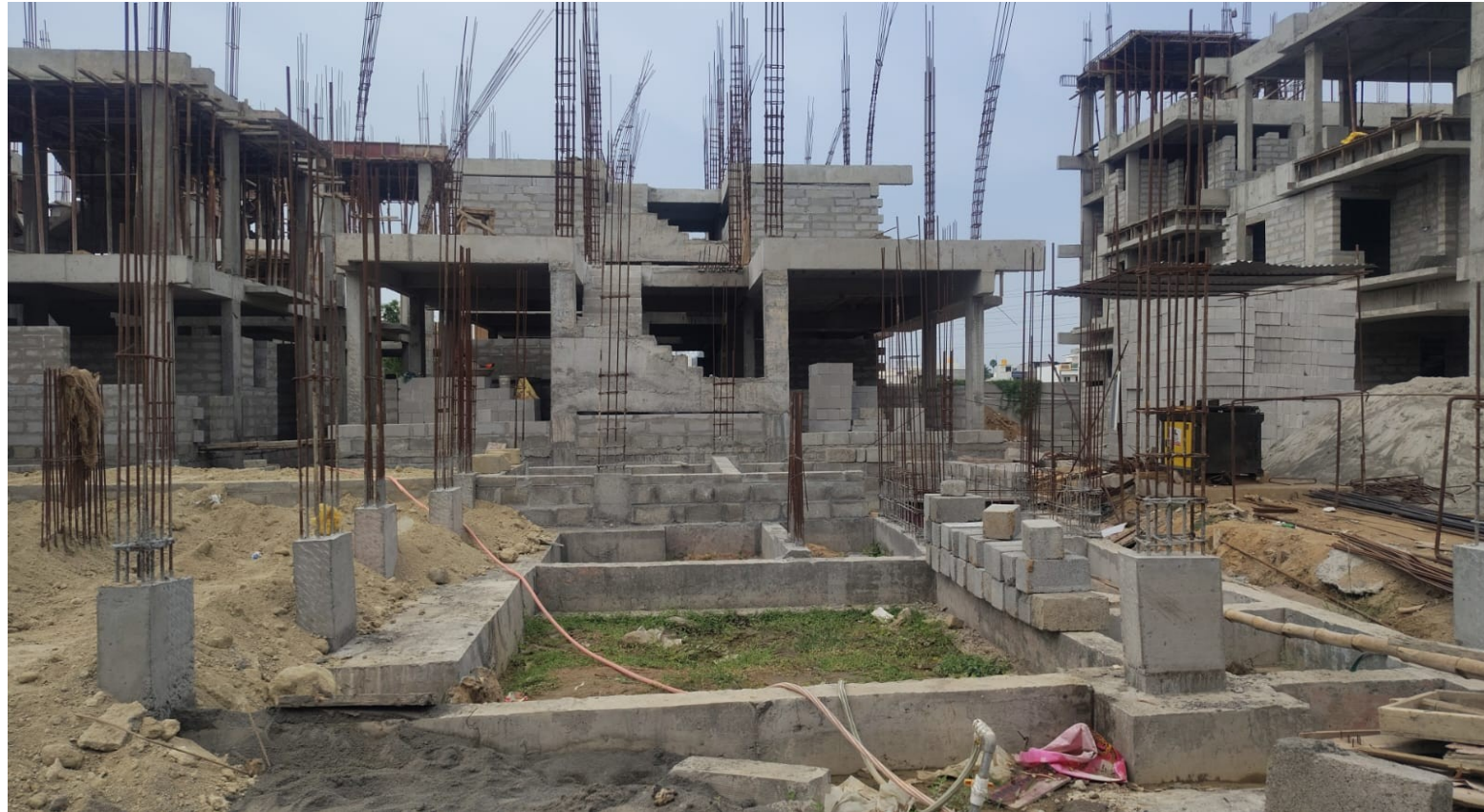
Villa No 35 –Basement Column Concrete Pouring work Completed
