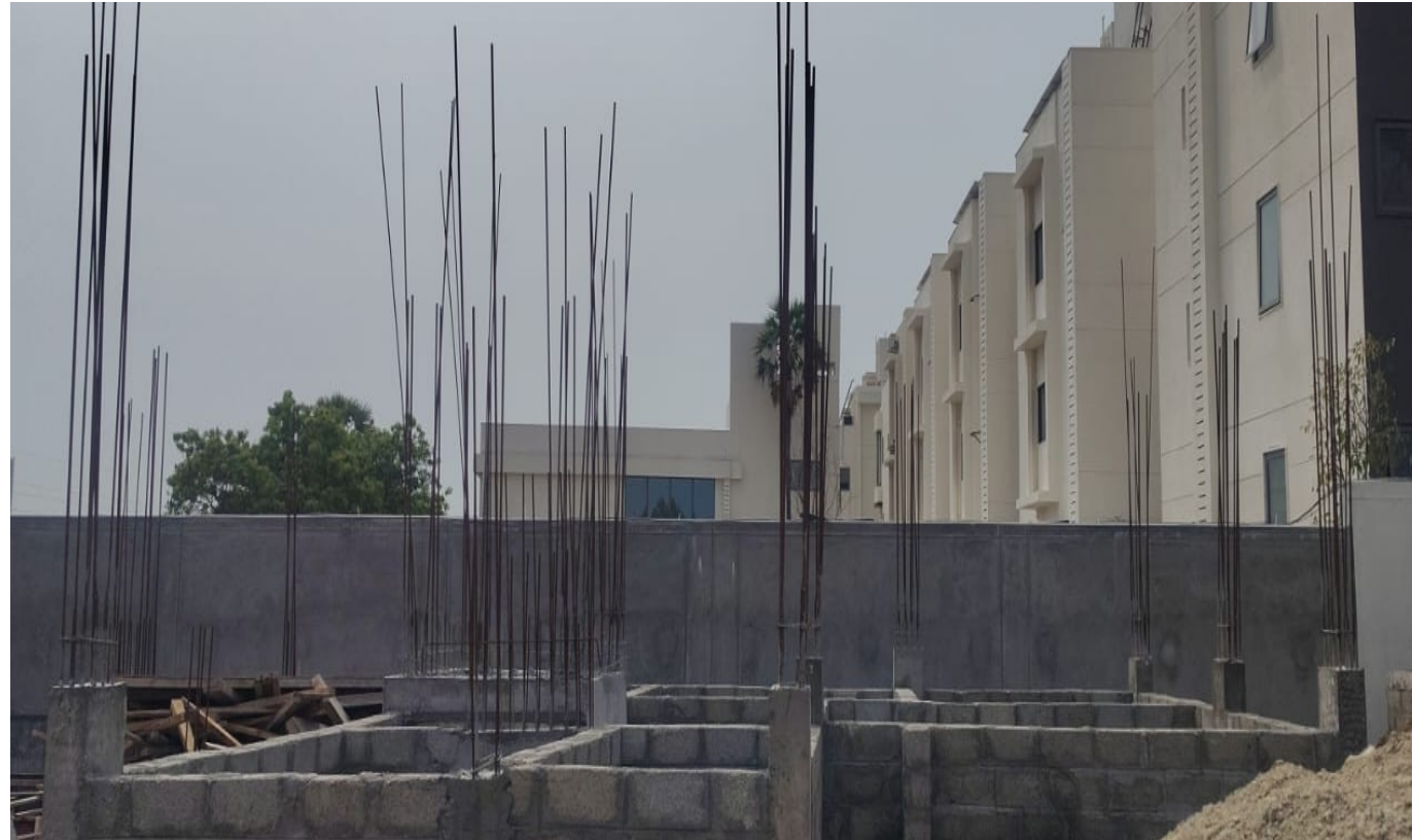
Villa No 122–Basement Block Work In Progress
