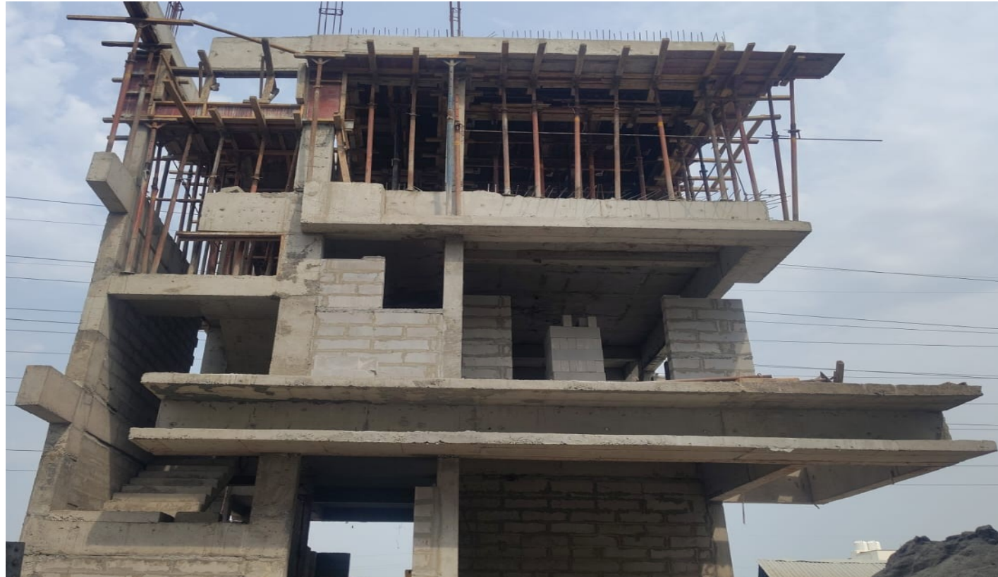
Villa No 46–FF Block Work In Progress
