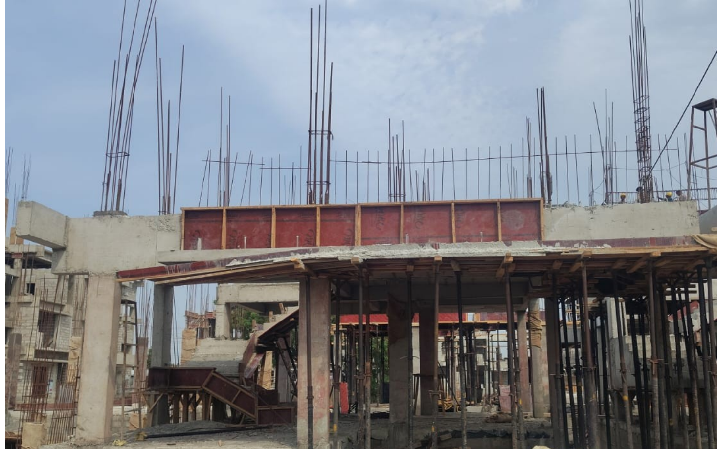
Villa No 118-FF Column Reinforcement Work Progress
