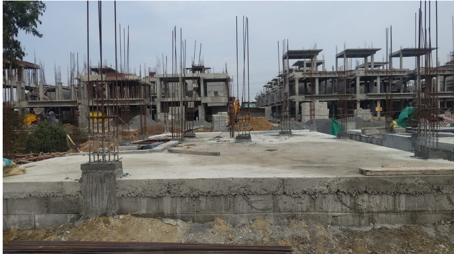
Villa No 111–GF Column Starter Concrete Completed
