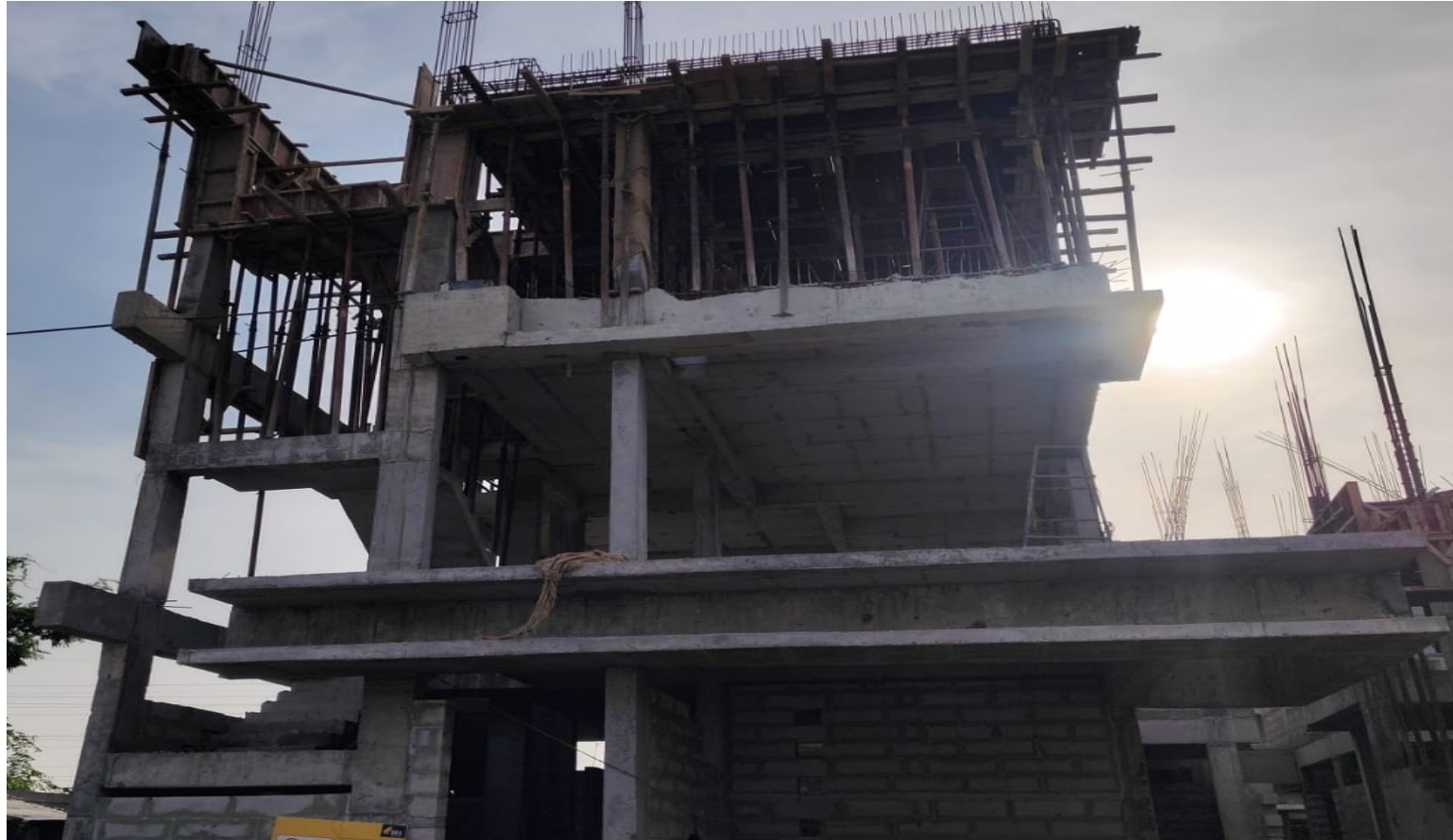
Villa No 30 – SF Roof Slab Reinforcement Work In Progress
