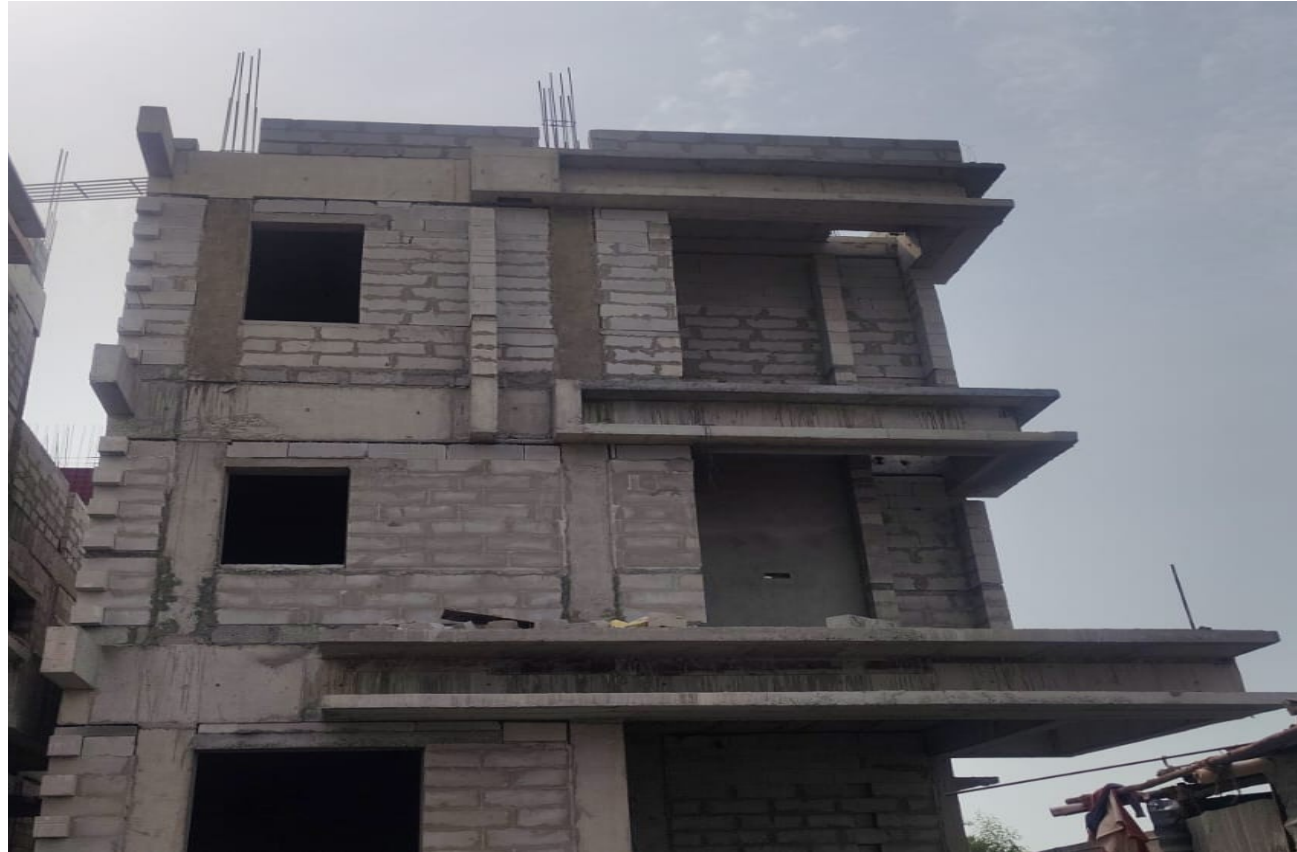
Villa No 45–Parapet Wall Block Work In Progress
