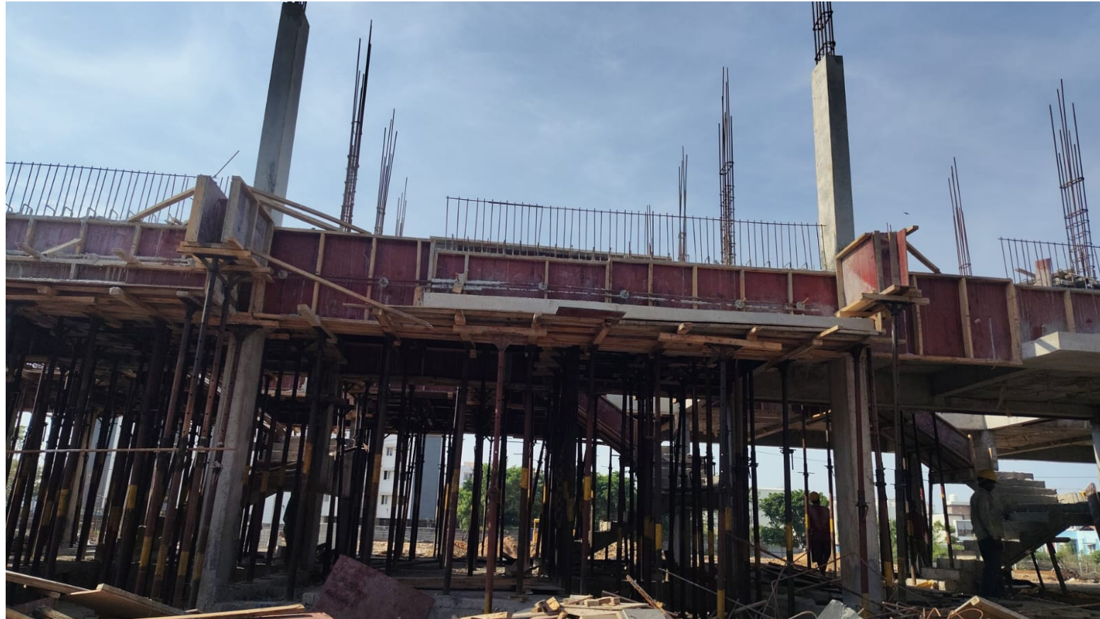
Villa No 91 To 96 –FF Column Concrete Pouring Completed
