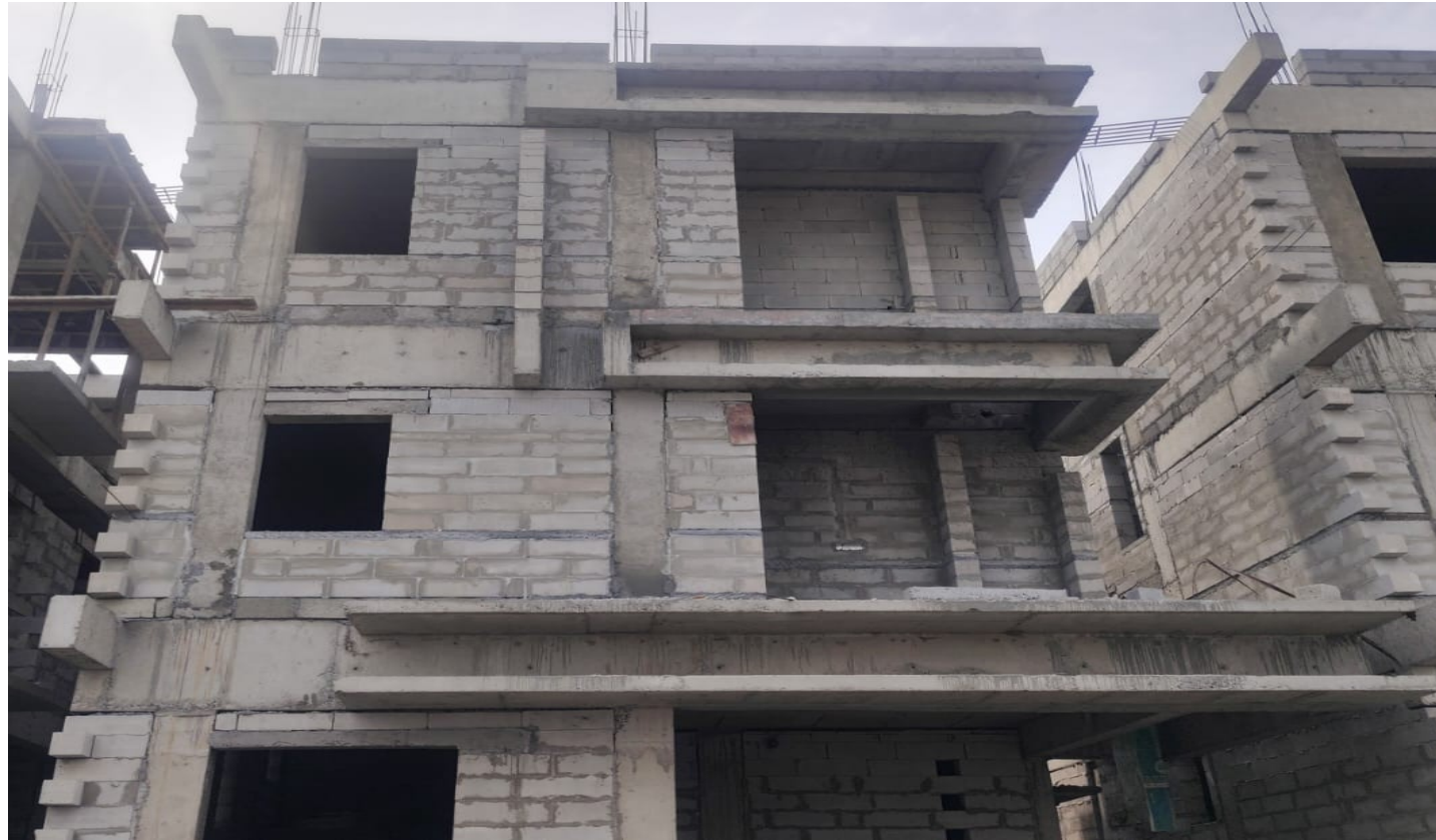
Villa No 44 –Parapet Wall Block Work In Progress
