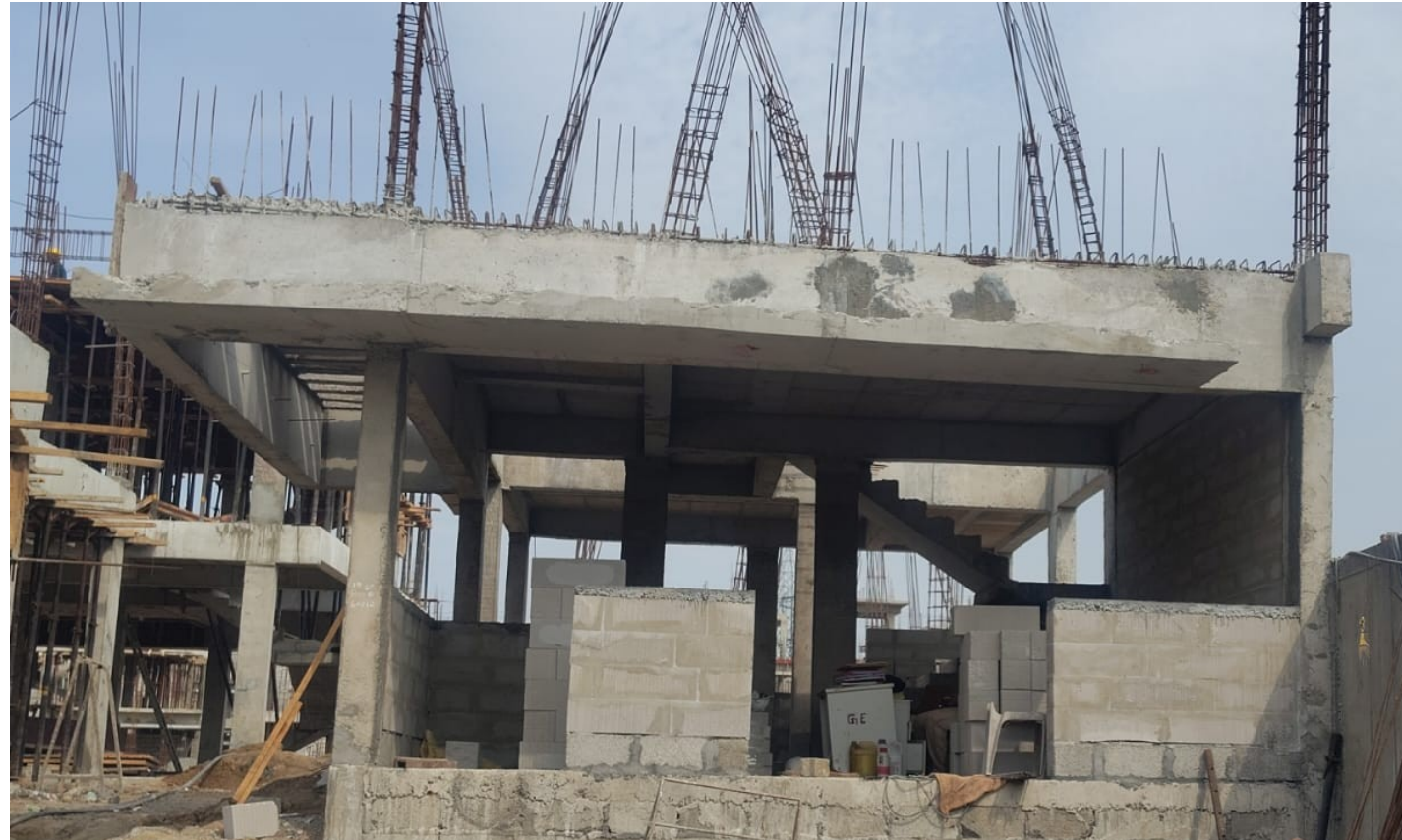
Villa No 120–GF Block Work In Progress
