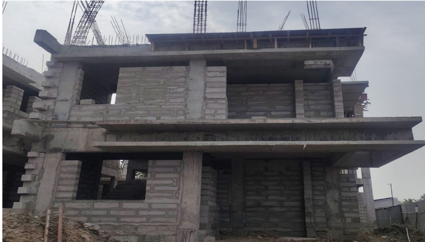
Villa No 38–FF Block Work In Progress
