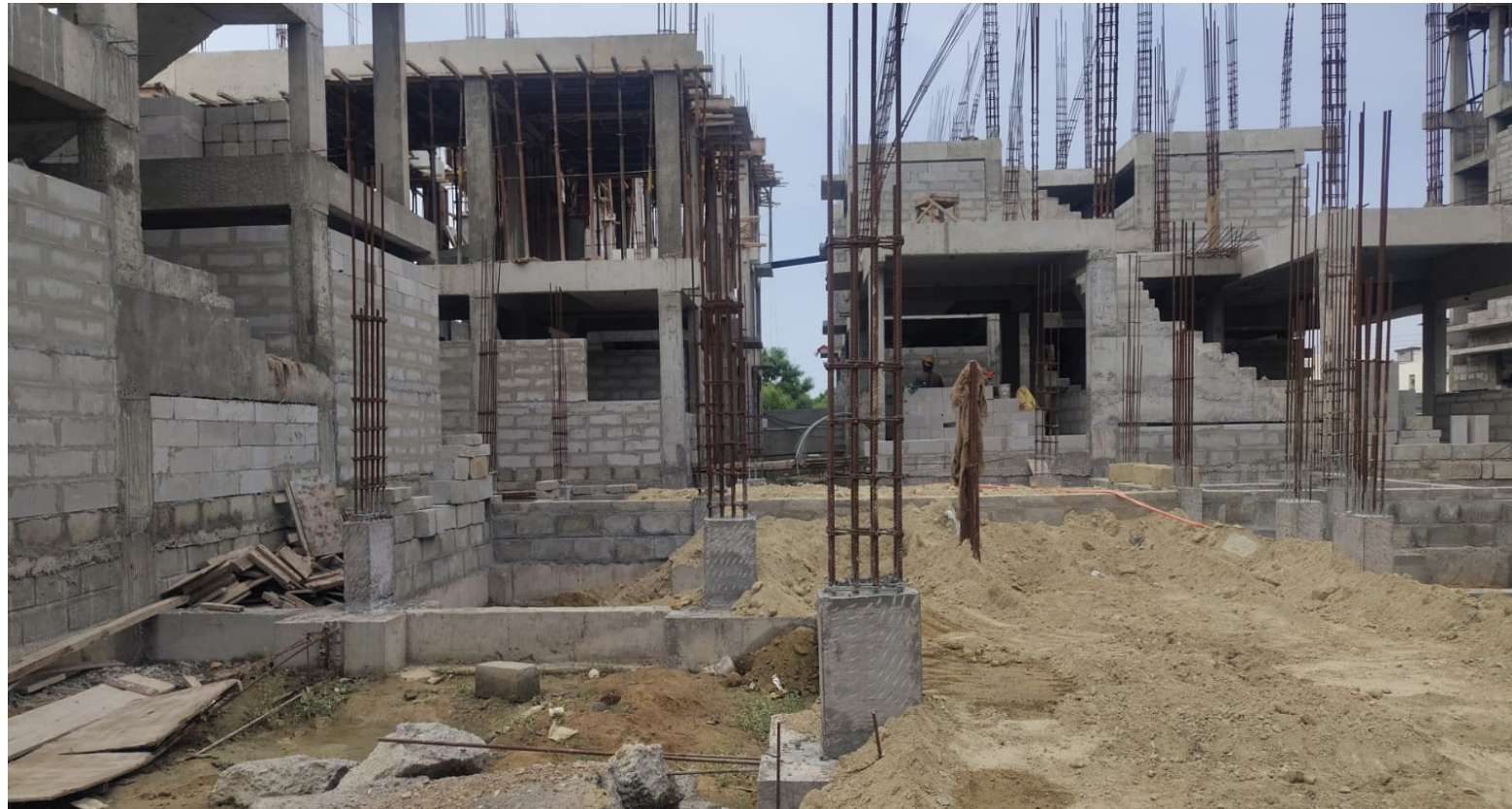
Villa No 34 –Basement Back Filling work In Progress
