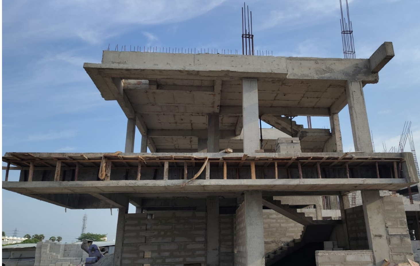
Villa No 33- FF Roof Slab Concrete Pouring work Completed
