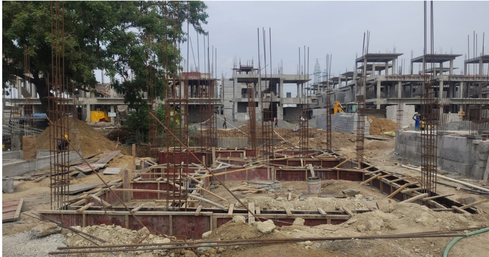
Villa No 110–Plinth Beam Shuttering Work In Progress
