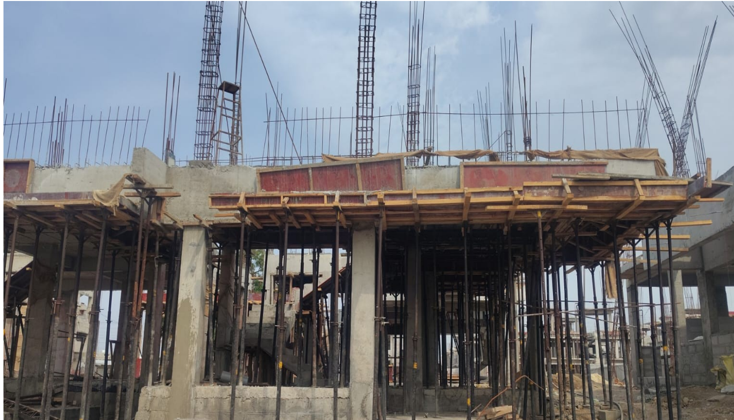
Villa No 119-FF Column Reinforcement Work Completed
