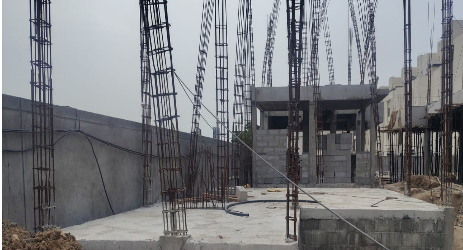
Villa No 113–GF Column Reinforcement Work Completed
