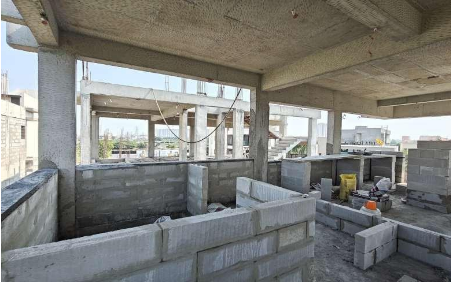
Villa No 4 – SF Bedroom blockwork in progress
