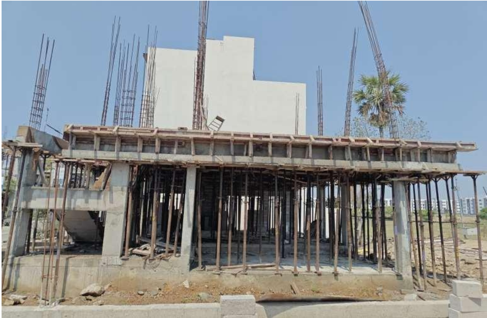
VillaNo 17 – GF Roof Slab Concreting work completed
