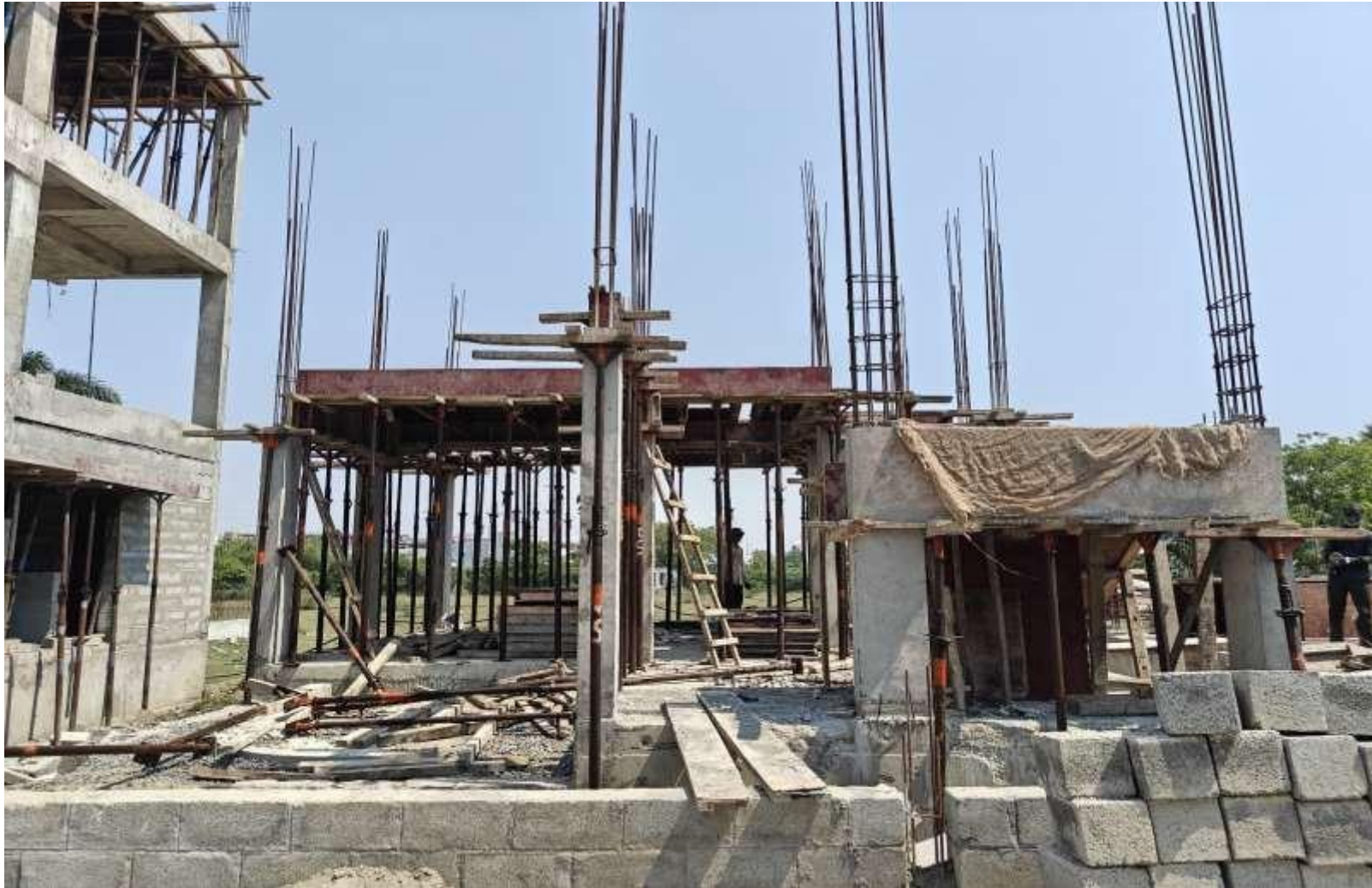
Villa No 13 – GF Roof Slab Shuttering work in progress
