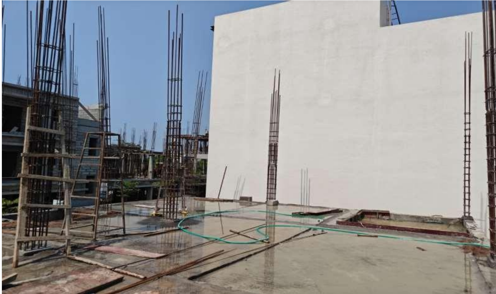
VillaNo 17 – FF Column Reinforcement work in progress
