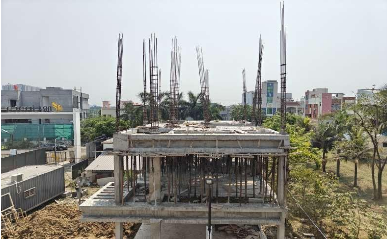
Villa No 3 – SF Column Reinforcement work in progress
