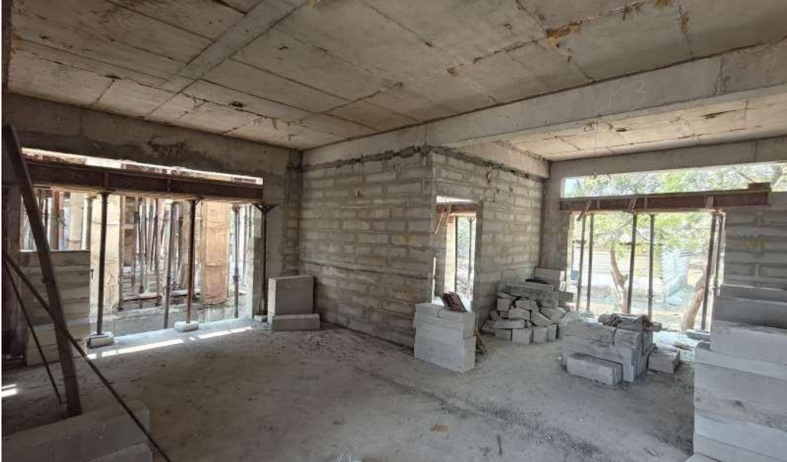
VillaNo 9 – Ground Floor Block work in progress
