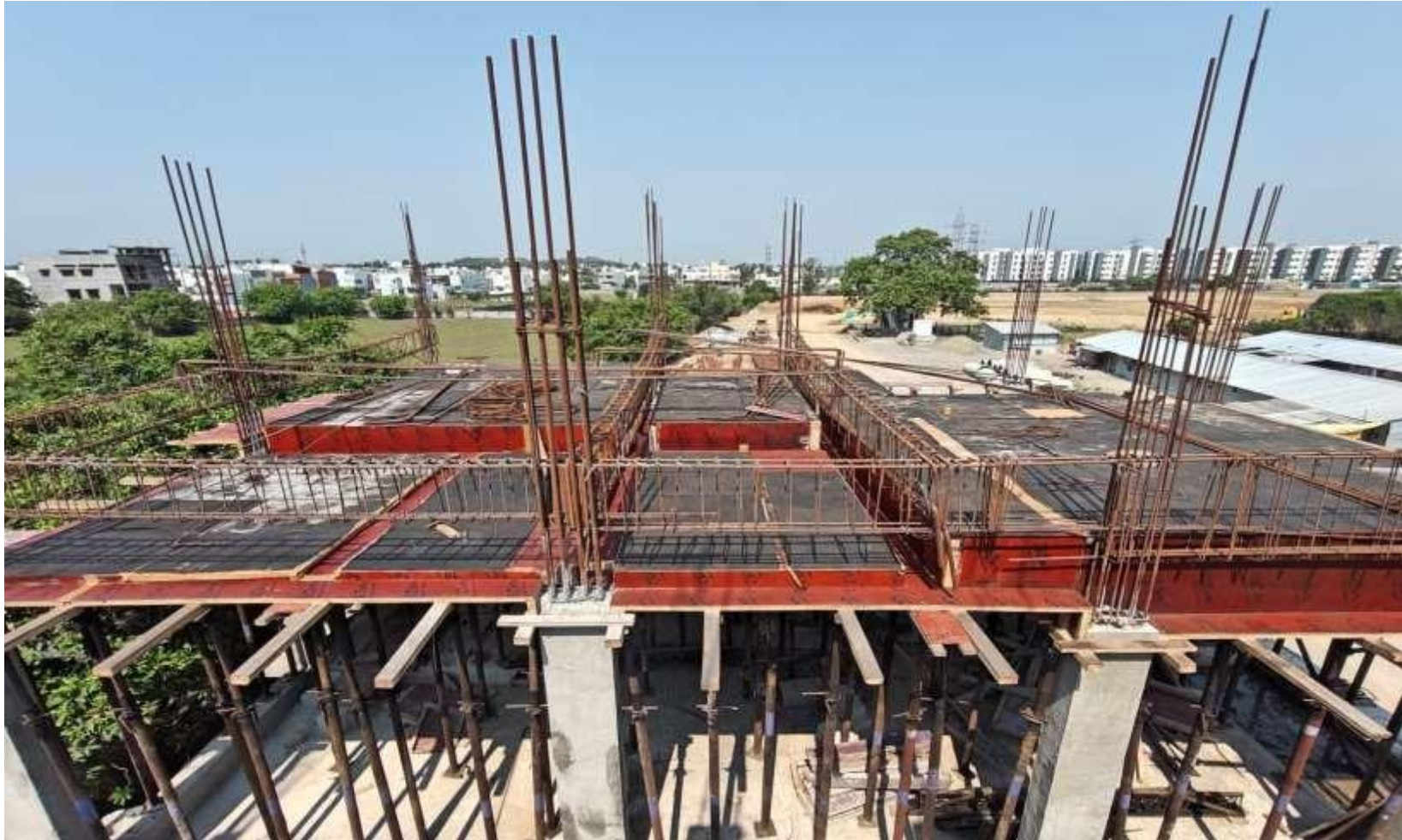
VillaNo 11 – FF Roof Slab Reinforcement Work in Progress
