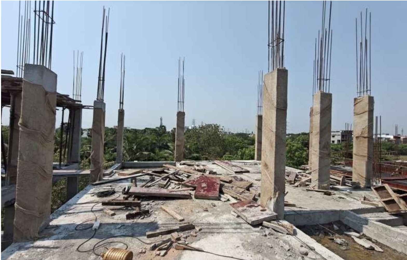
Villa No 10 – SF Column concreting work completed
