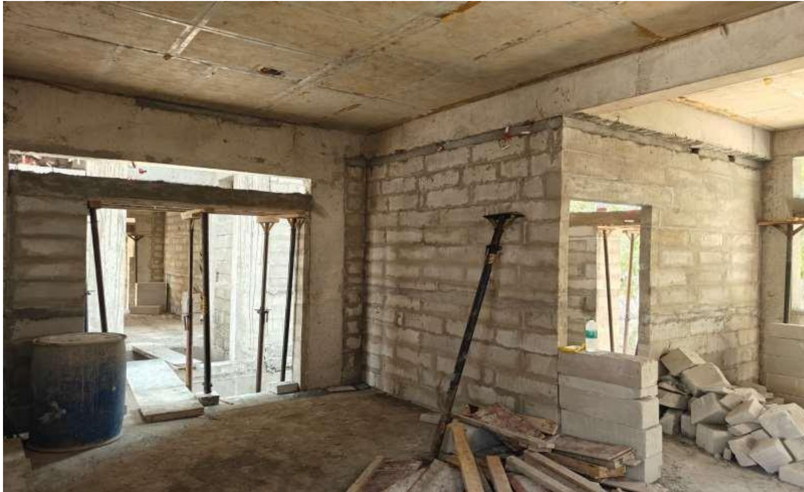
VillaNo 11 – GF LivingBlock work in Progress
