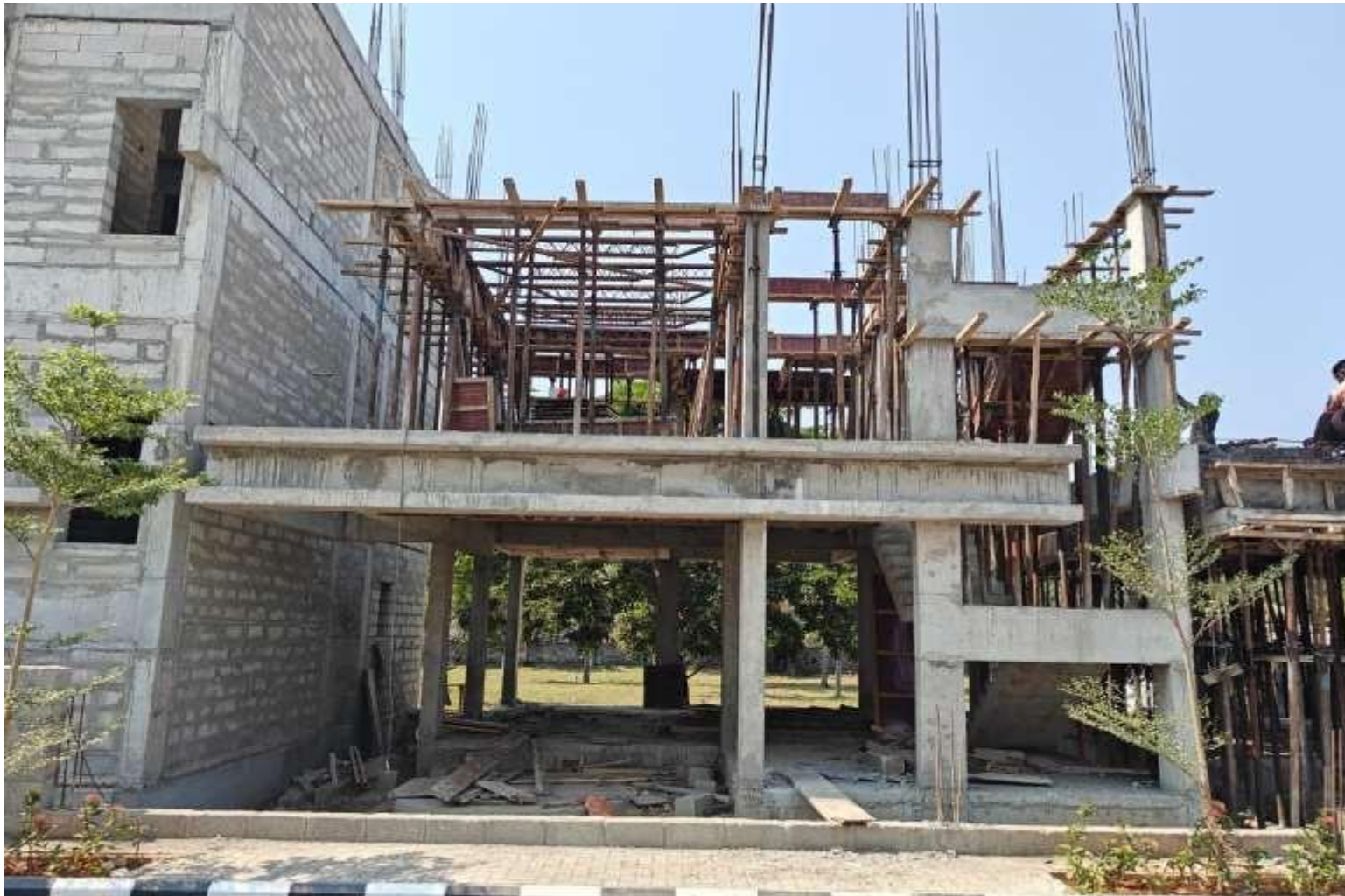
VillaNo 07– FF Roof slab Shuttering work in progress
