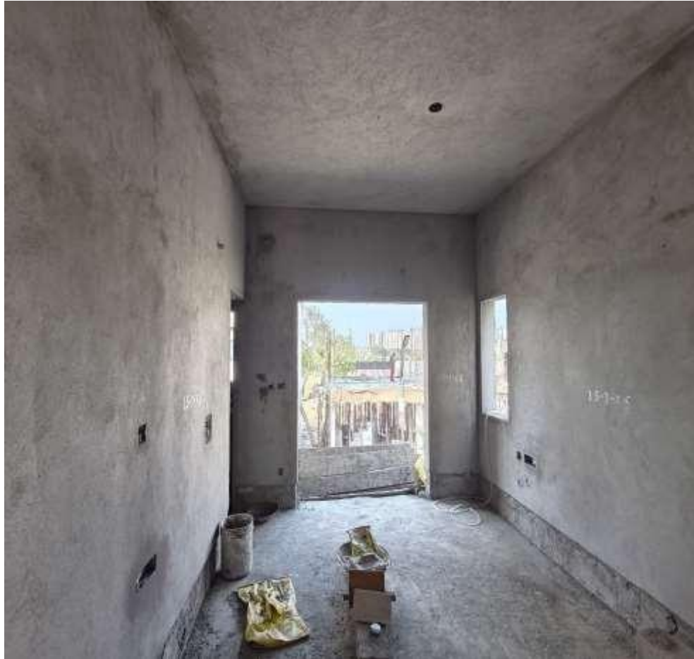
Villa -6 FF Bedroom- 1&2 Internal Wall Plastering work in progress
