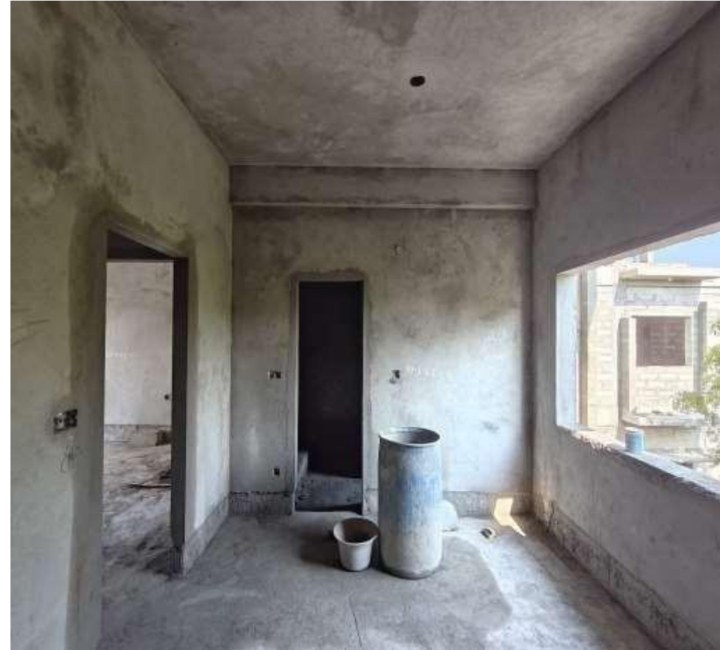
Villa -6 FF Bedroom- 1&2 Internal Wall Plastering work in progress
