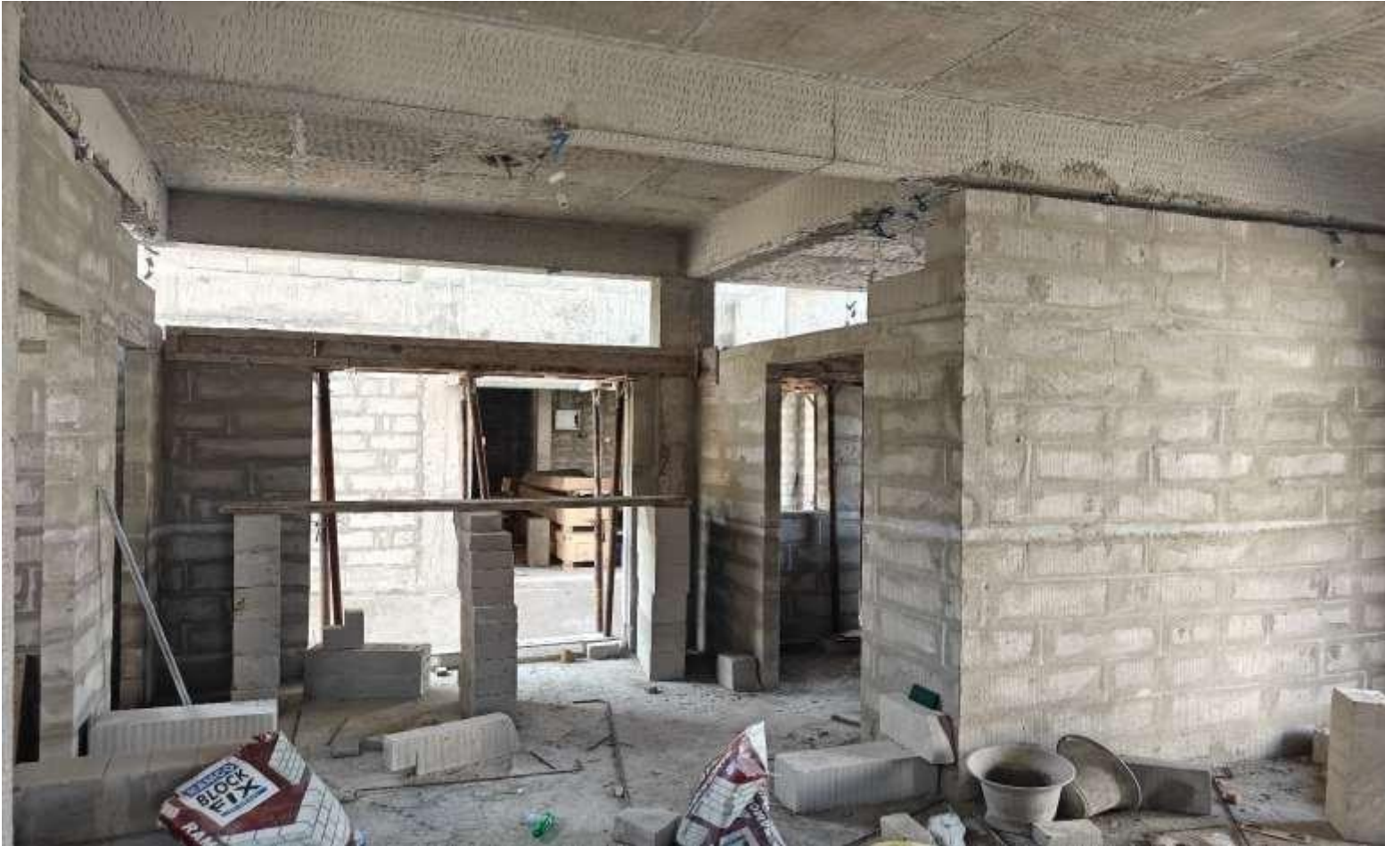
VillaNo5 – Ground Floor Blockwork in Progress
