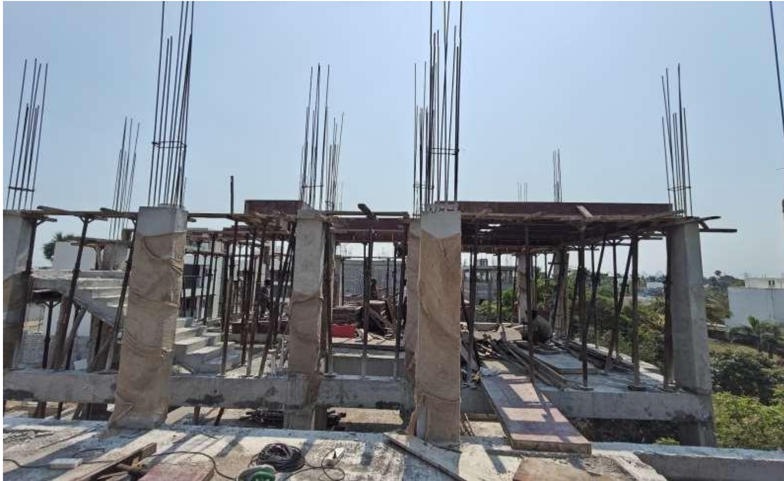
VillaNo 09 – SF Roof Slab Shuttering Work in progress
