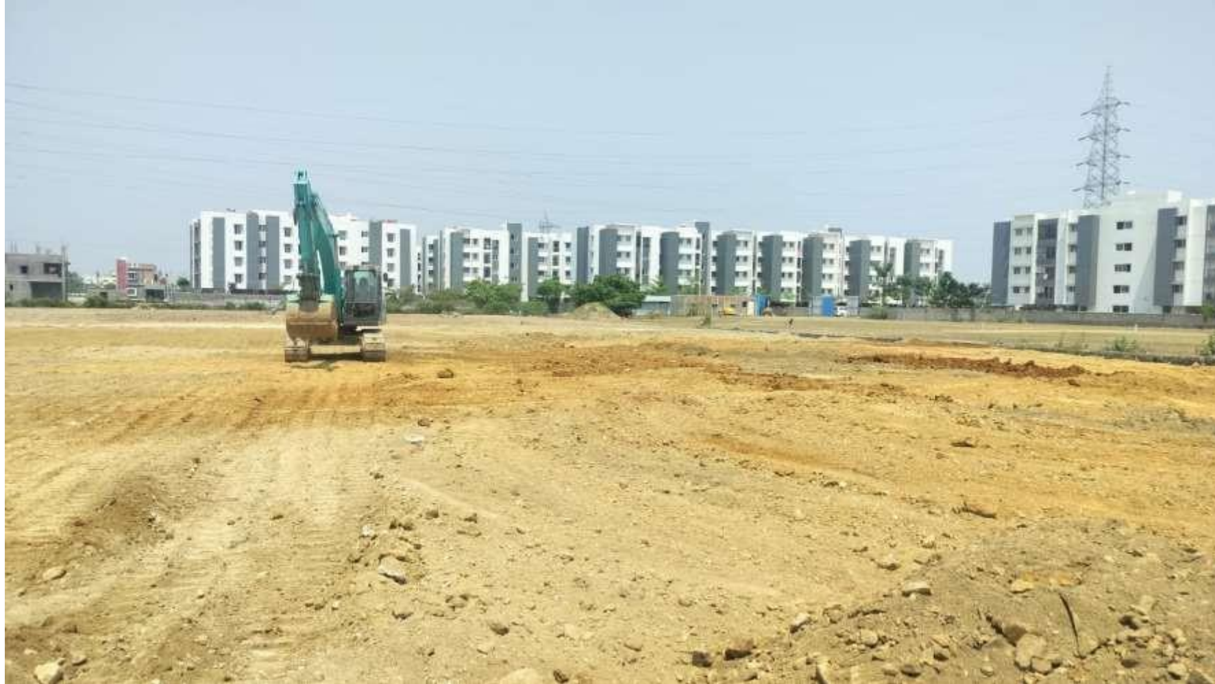
Phase-2 Soil Filling and Levelling work in Progress
