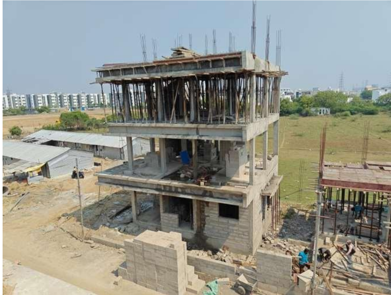
Villa No 12– SF Roof Slab Concreting Work Completed
