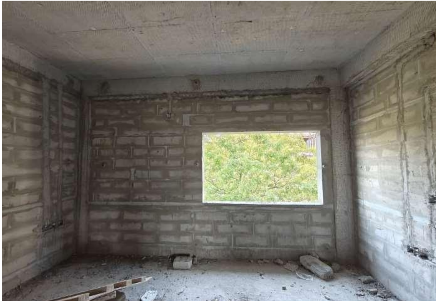
Villa No 4 – FF Bedroom Electrical pipeline laying work in progress
