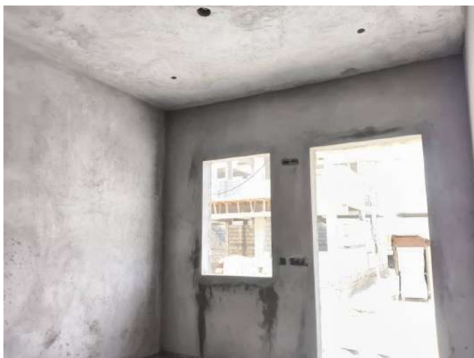
V64 - Internal Plastering
