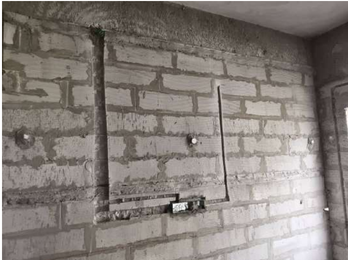
V42 - Instllation of Wall chasing & Electrical conduits
