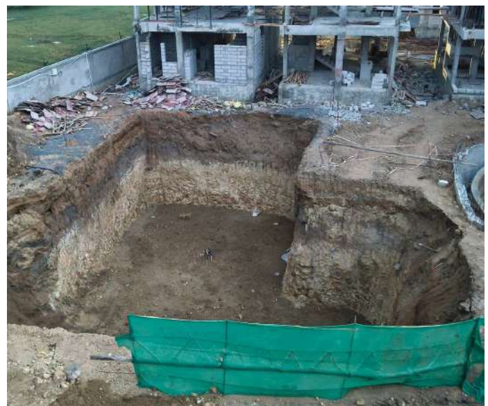
STP - Civil works
