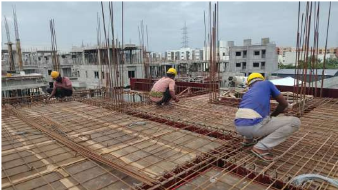
V113 - First Floor Roof Slab & Beam - Shuttering, Reinforcement
