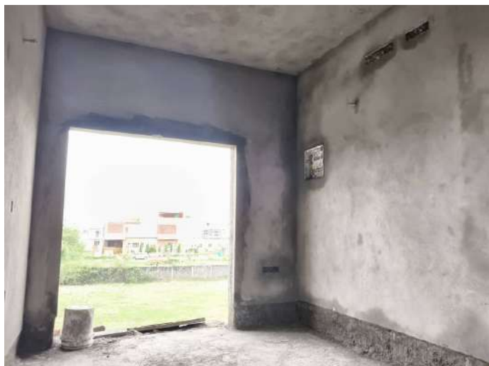
V38 - Internal Plastering
