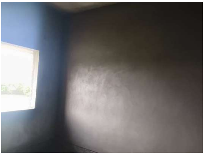
V29 - Internal Plastering
