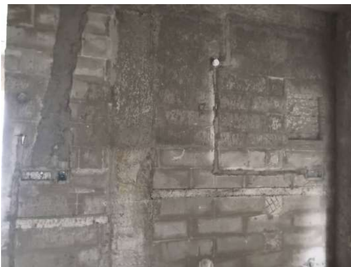
V52 - Instllation of Wall chasing & Electrical conduits
