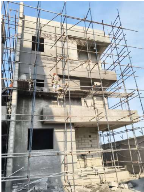
V45 - External Plastering
