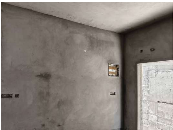
V65 - Internal Plastering
