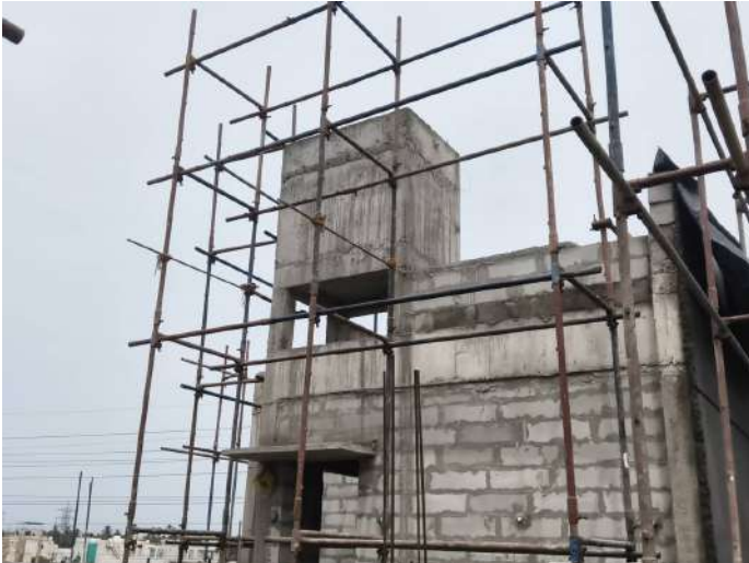
V45 - OHT Cover Slab Concreting
