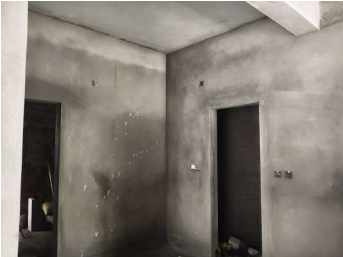
V42 - Internal Plastering
