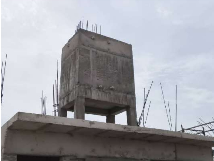
V43 - OHT Cover Slab Concreting
