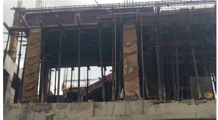
V115 - First Floor Column Concreting
