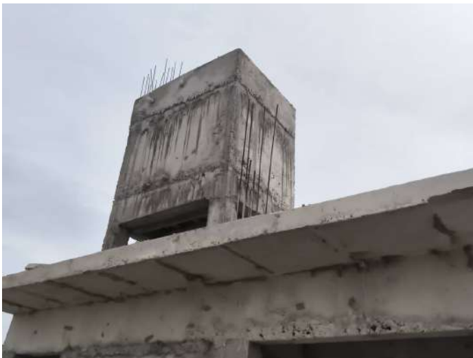
V42 - OHT Cover Slab Concreting
