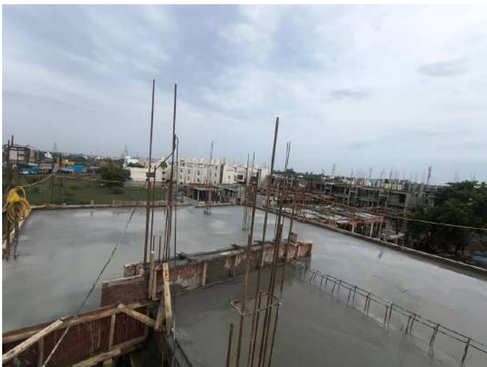
V108 - SF- Roof Slab & Beam Concreting
