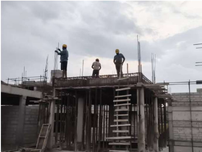
V36 - Stair Head Room Roof Slab & Beam - Shuttering, Reinforcement
