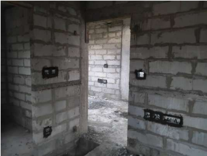
V33 - Instllation of Wall chasing & Electrical conduits
