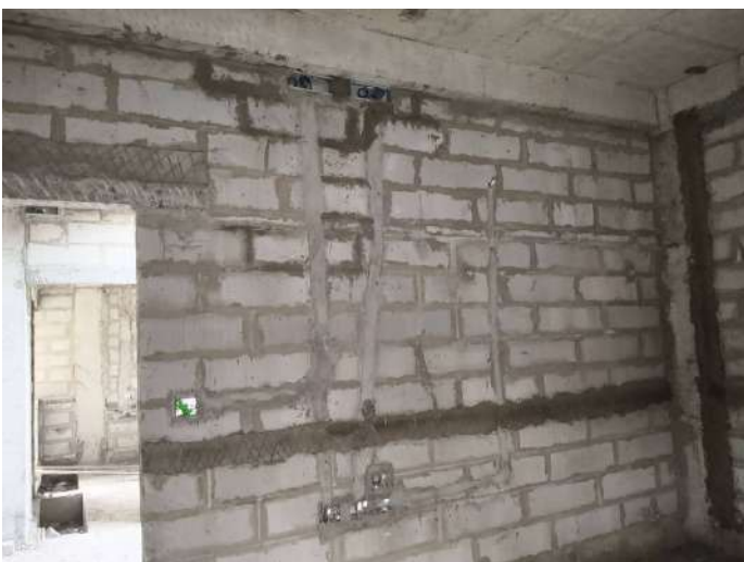
V37 - Instllation of Wall chasing & Electrical conduits
