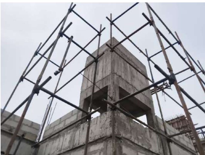
V40 - OHT Cover Slab Concreting
