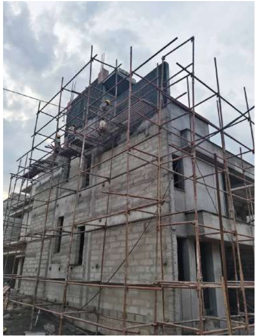
V71 - External Plastering
