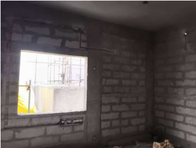
V42 - Instllation of Wall chasing & Electrical conduits
