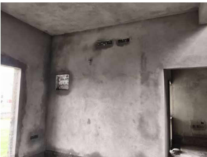
V38 - Internal Plastering
