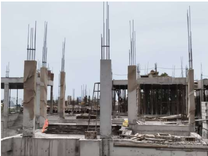
V36 - Stair Head Room Column Concreting
