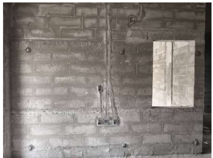
V52 - Instllation of Wall chasing & Electrical conduits
