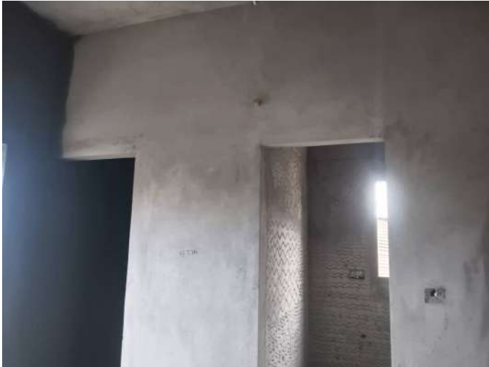
V29 - Internal Plastering
