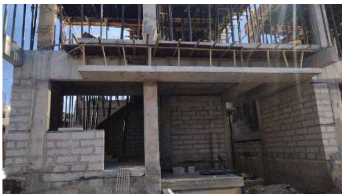
V118 - Completion of Ground Floor Roof Slab
