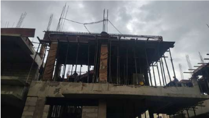
V115 - First Floor Roof Slab & Beam - Shuttering, Reinforcement
