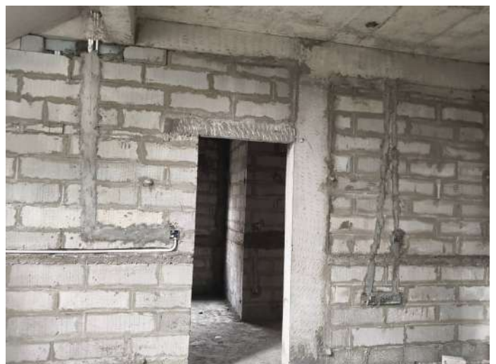
V37 - Instllation of Wall chasing & Electrical conduits
