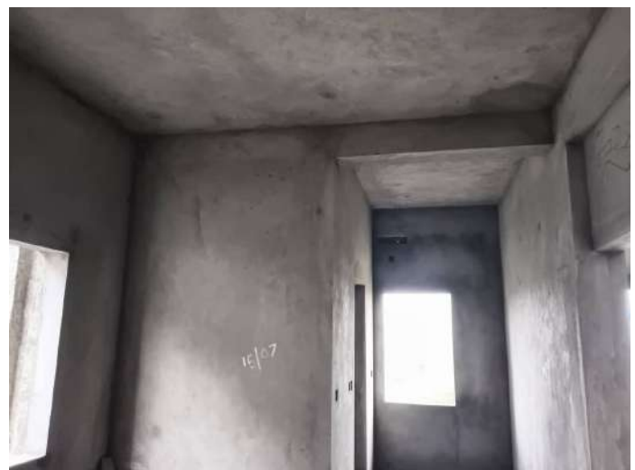
V38 - Internal Plastering
