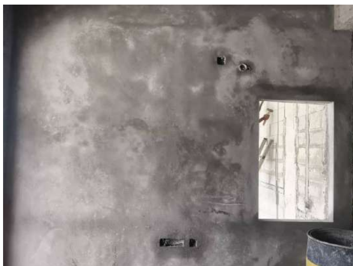
V63 - Internal Plastering
