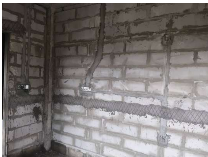
V38 - Instllation of Wall chasing & Electrical conduits
