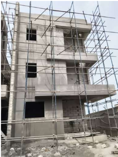
V45 - External Plastering
