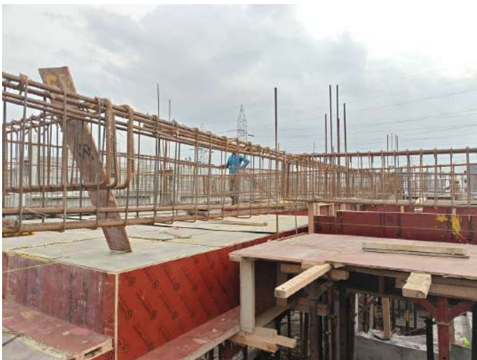
V92 - First Floor Roof Slab & Beam - Shuttering, Reinforcement
