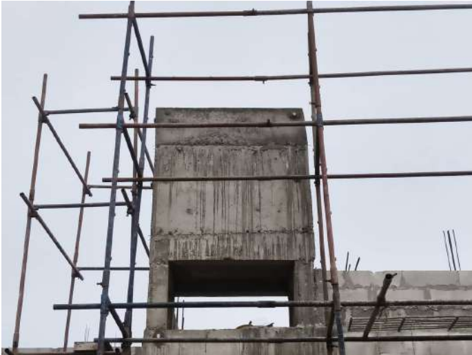
V44 - OHT Cover Slab Concreting
