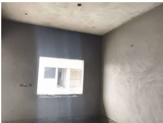
V37 - Internal Plastering
