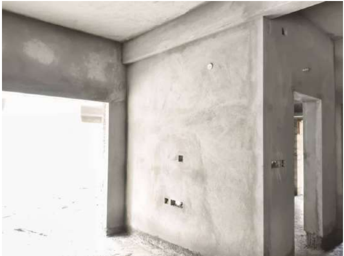
V42 - Internal Plastering
