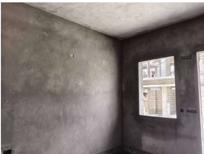
V65 - Internal Plastering
