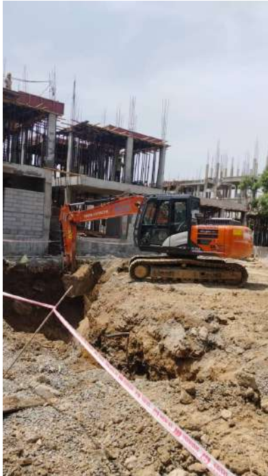
STP - Civil works
