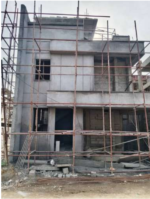
V71 - External Plastering
