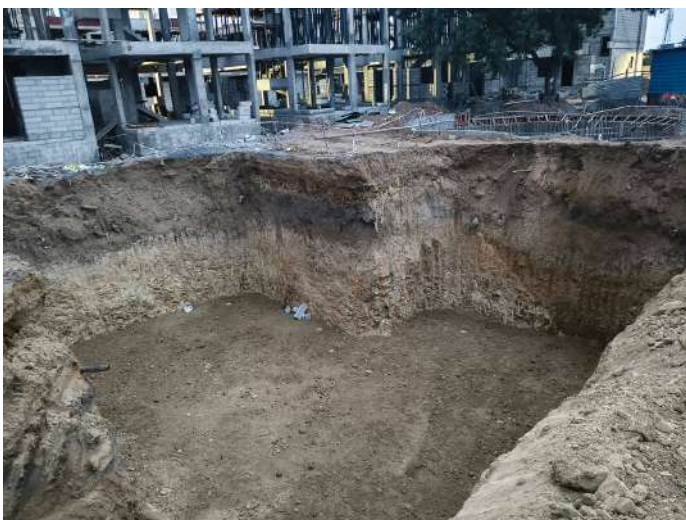
STP - Civil works
