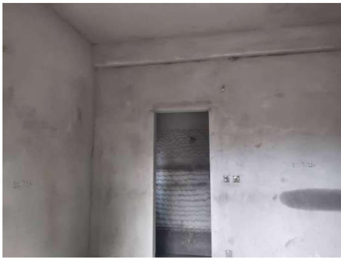
V29 - Internal Plastering
