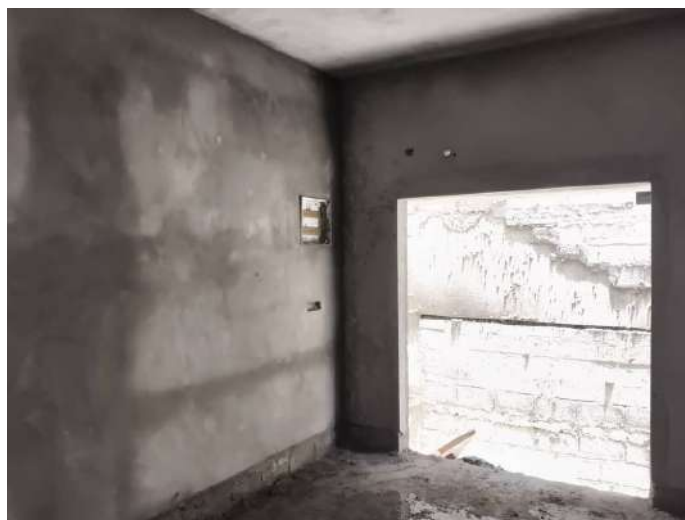
V64 - Internal Plastering
