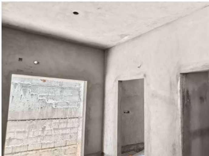
V65 - Internal Plastering
