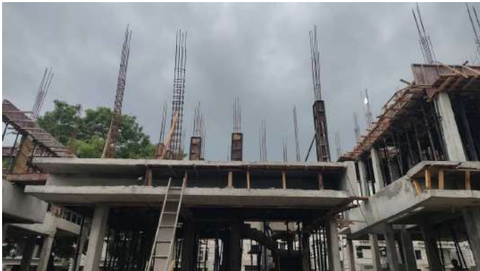
V110 - First Floor Column Concreting
