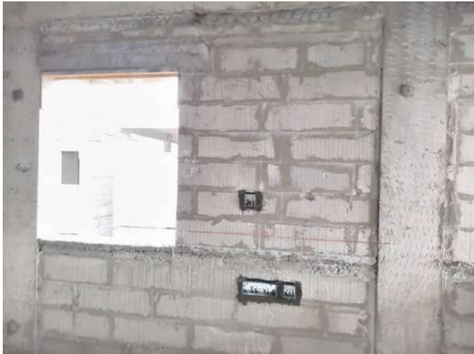
V33 - Instllation of Wall chasing & Electrical conduits
