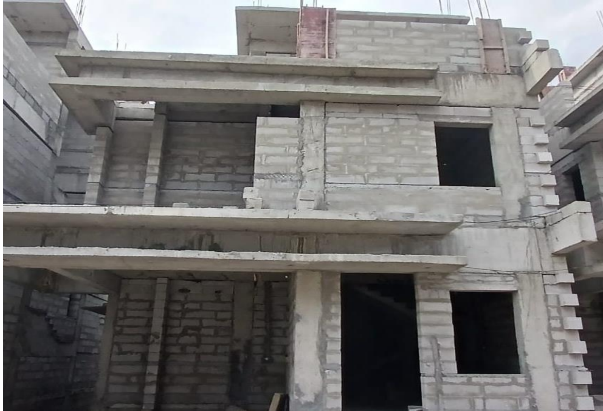
Villa No 66–Parapet Wall Block Work In Progress
