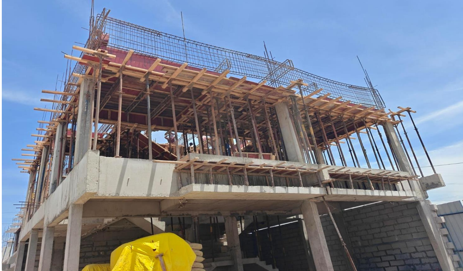
Villa No 97 to 98–FF Roof Slab Beam Reinforcement Work In Progress
