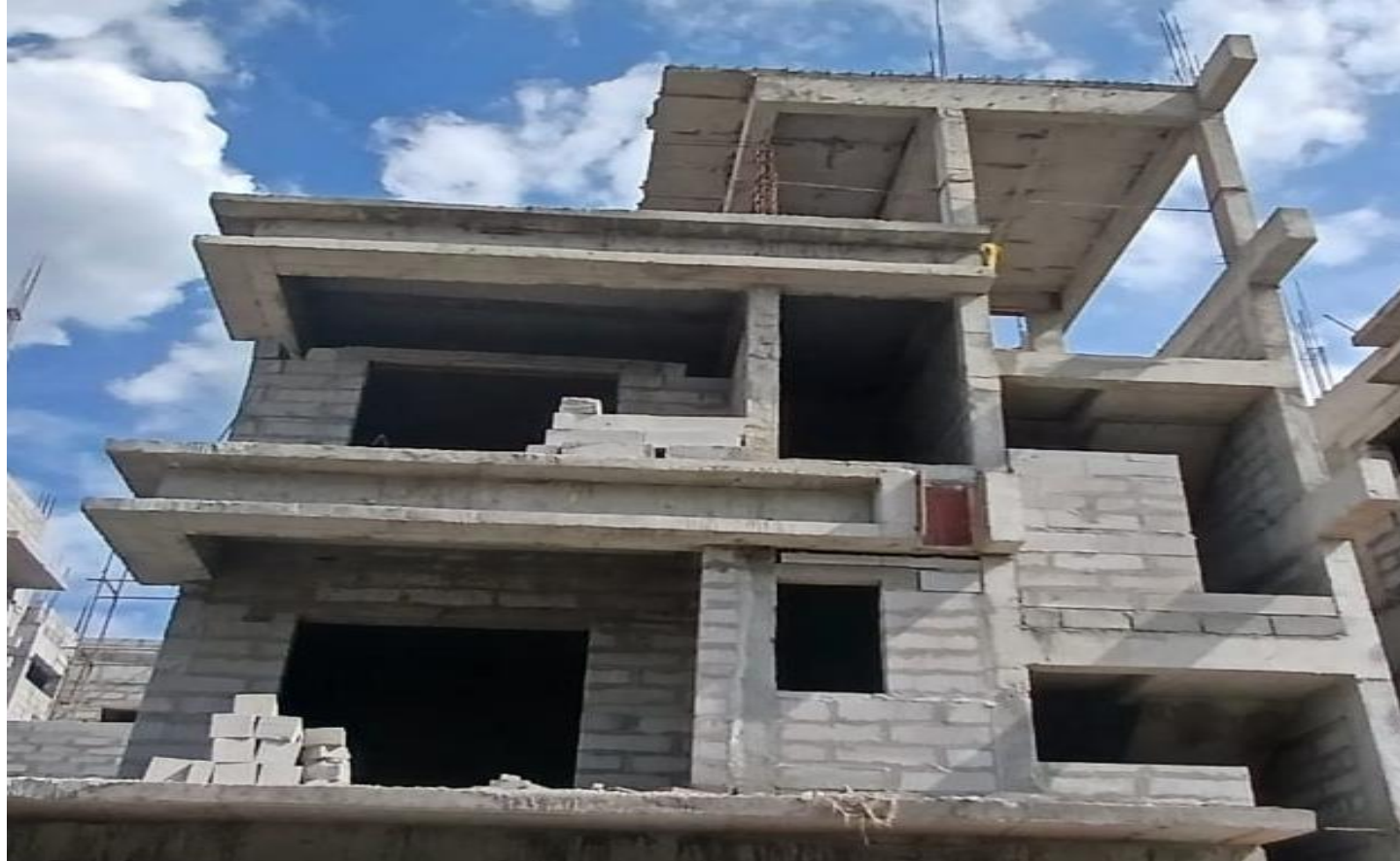
Villa No 42 – SF Block Work In Progress
