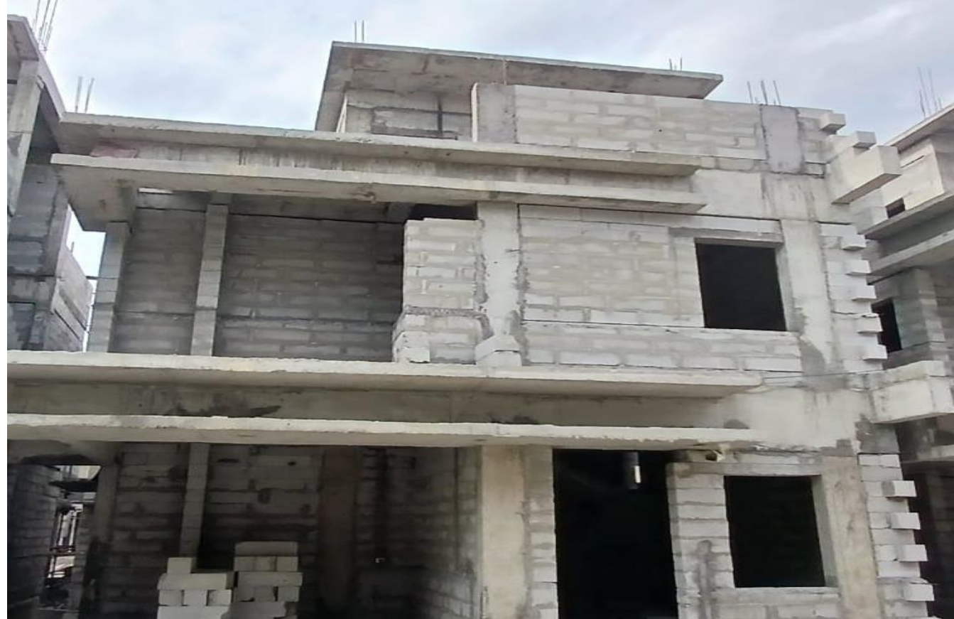
Villa No 67 –Parapet Wall Block Work In Progress
