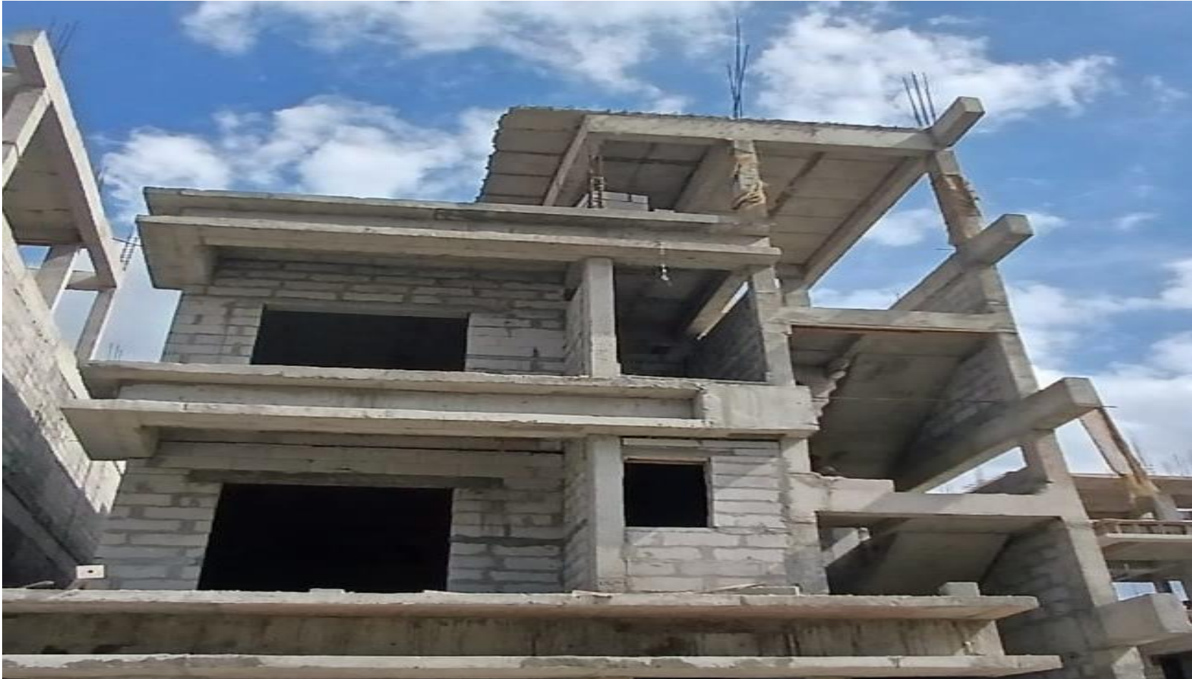
Villa No 43- SF Block Work In Progress
