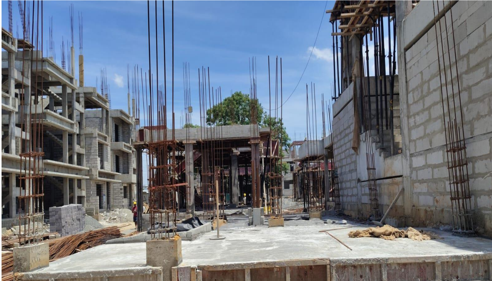
Villa No 117–GF Floor PCC Concrete Pouring Completed
