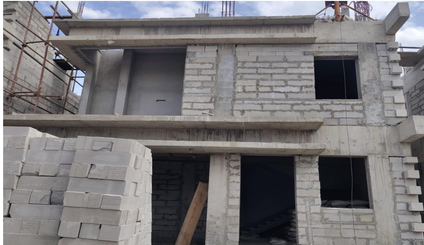
Villa No 77 –FF Plastering Work In Progress
