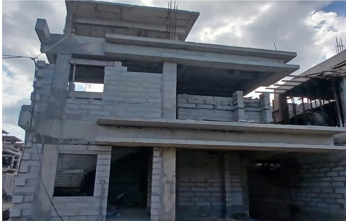
Villa No 71 –FF Block Work In Progress
