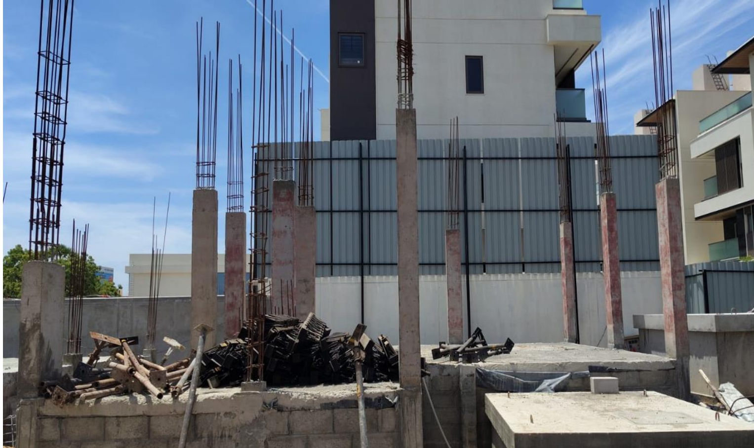
Villa No 123–GF Colum Concrete Pouring Work Completed
