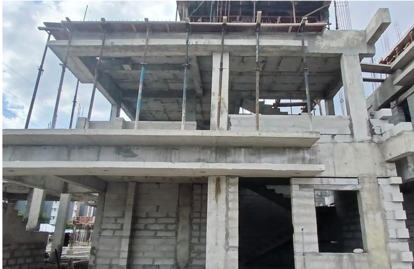
Villa No-63 FF Block Work In Progress
