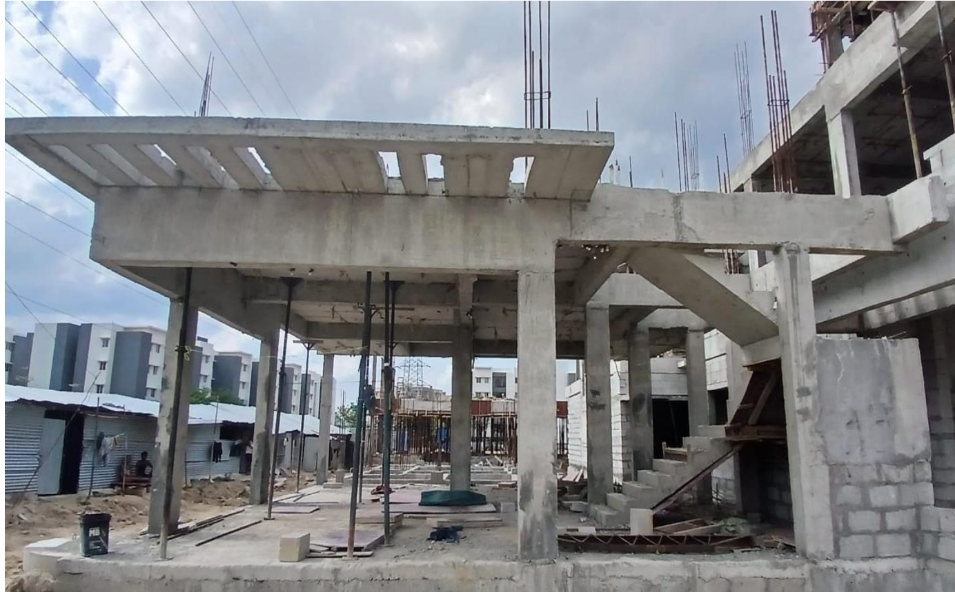
Villa No 62-GF Roof Slab Concrete Pouring Completed
