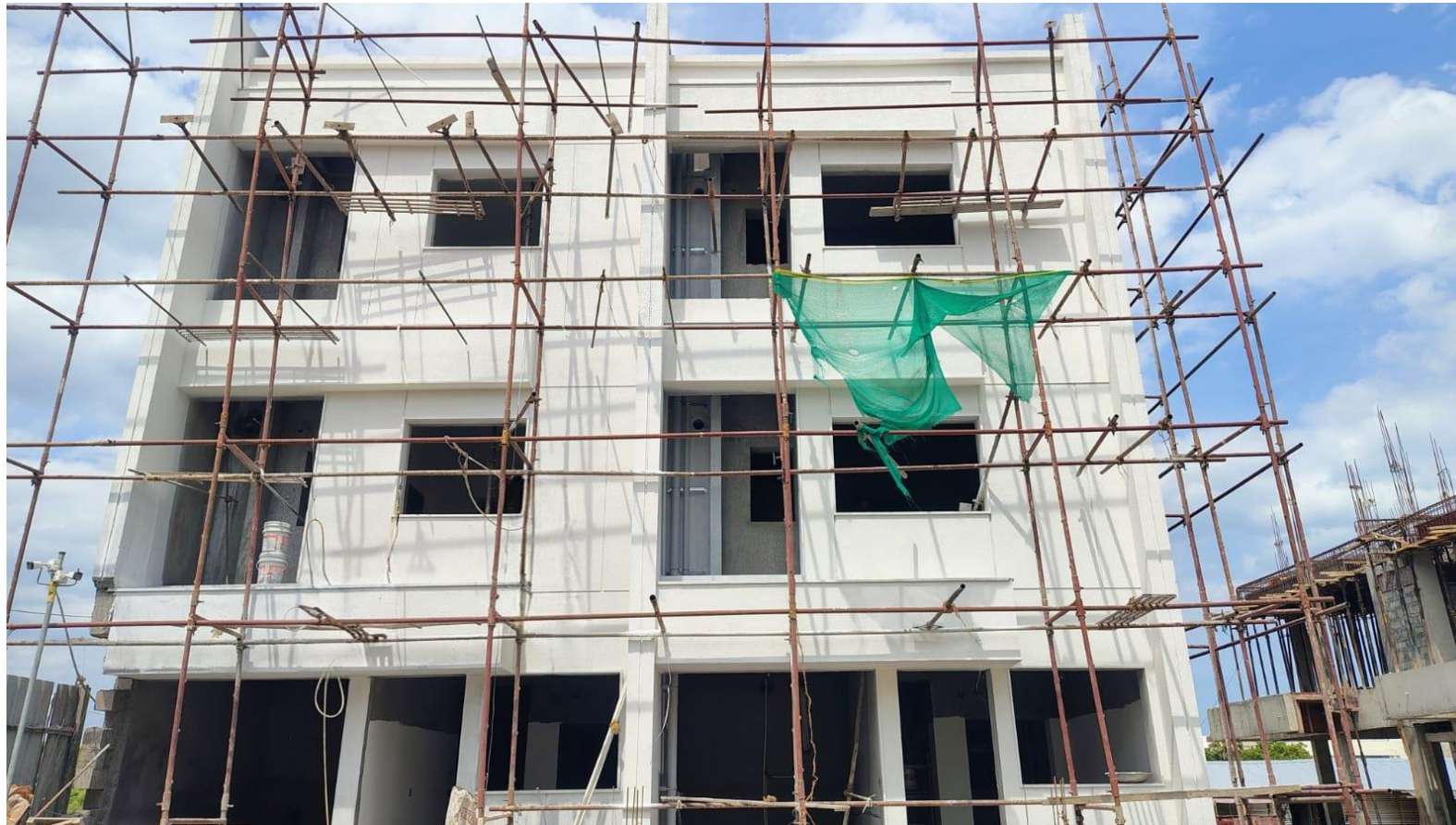
Villa No 99 to 100–External Texture Painting Work In Progress
