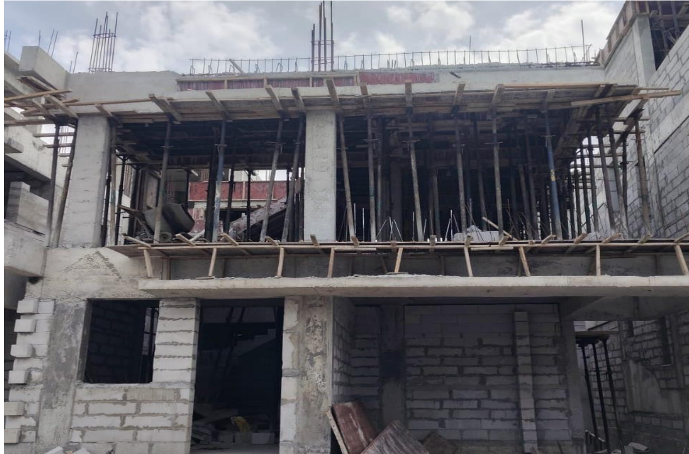
Villa No 72 –GF Block Work Completed
