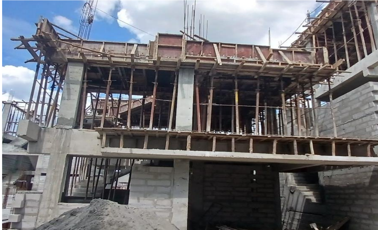
Villa No 36–FF Roof Slab Concrete Pouring Work Completed
