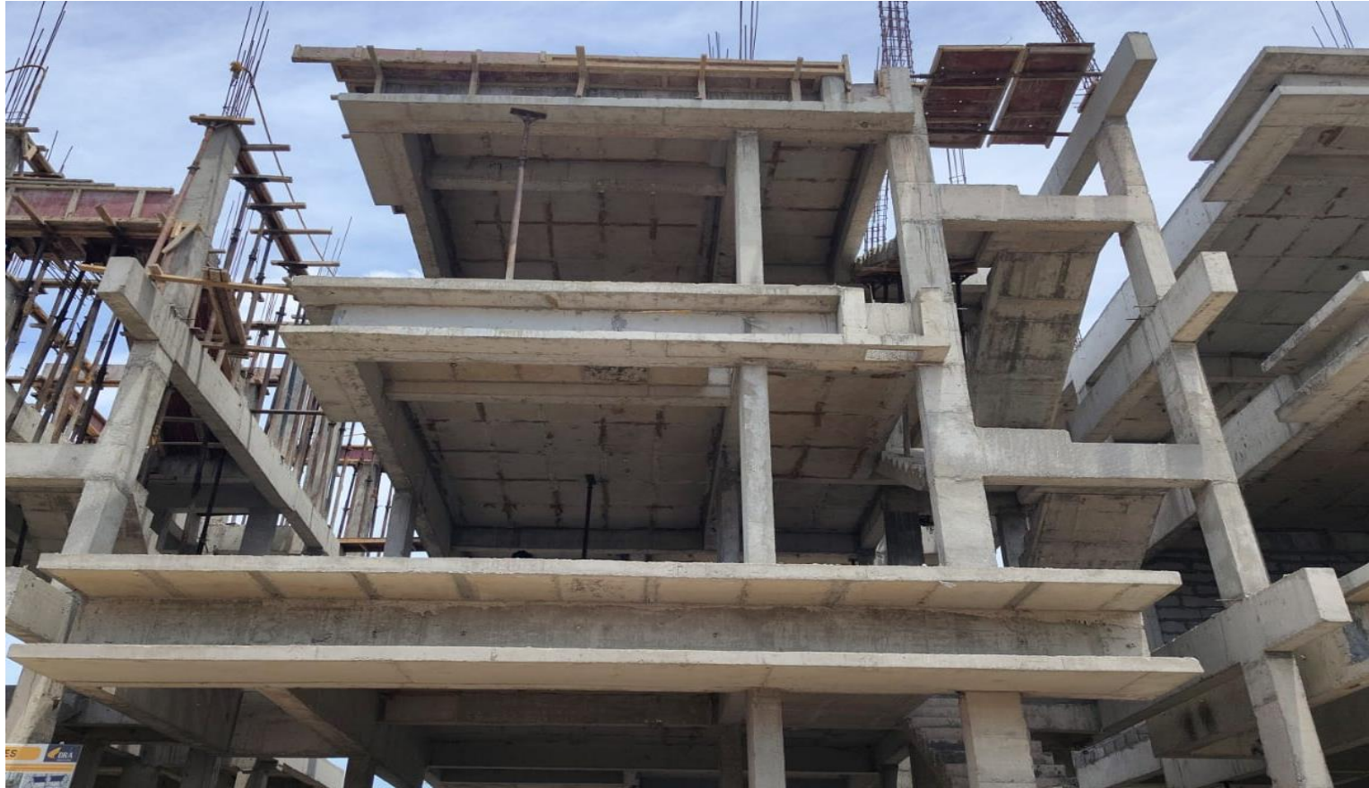
Villa No 26- Head Room Column Reinforcement Work In Progress
