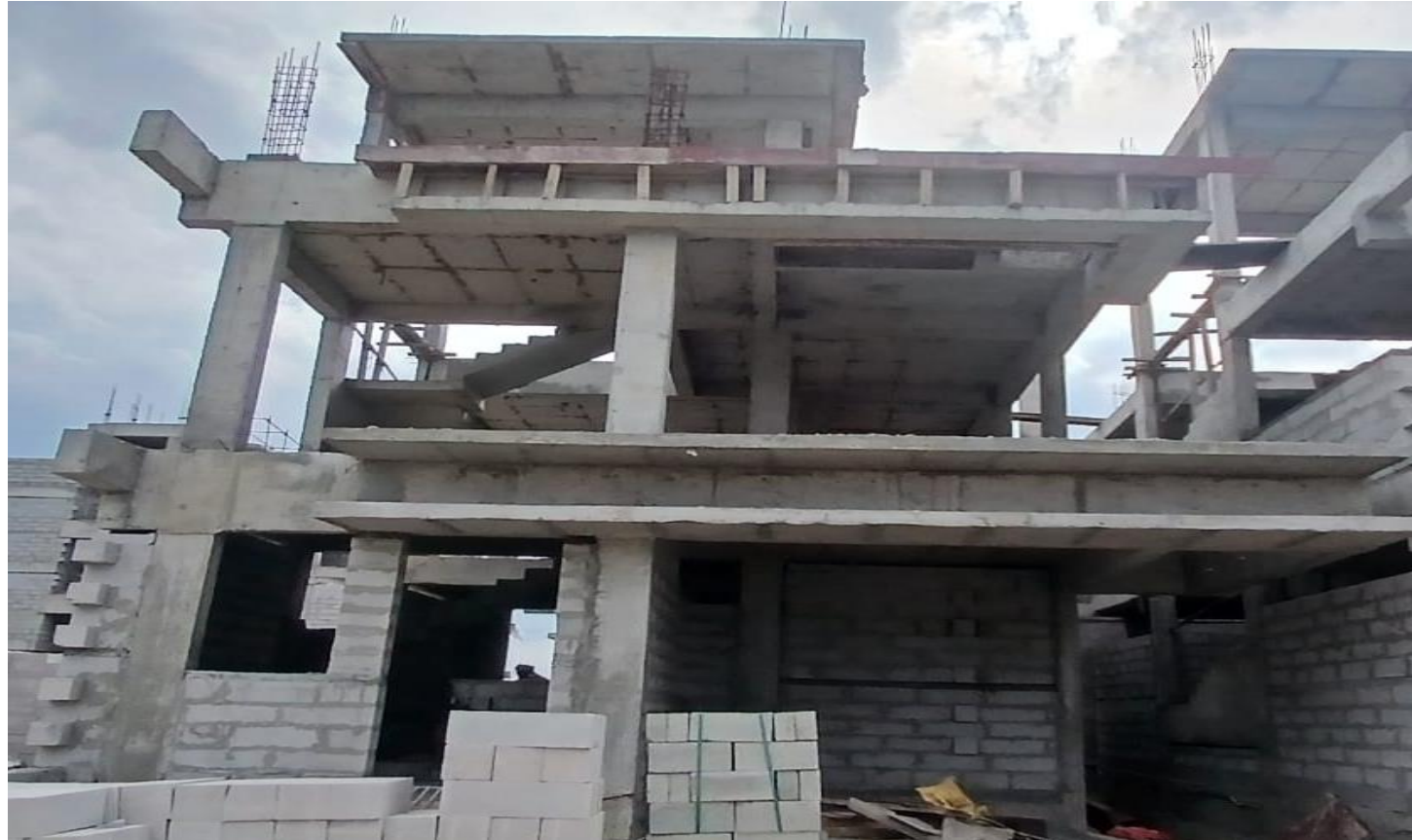
Villa No-53 GF Block Work Completed
