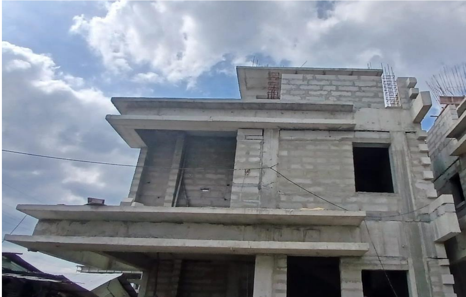
Villa No 47 – Parapet Wall Block Work In Progress
