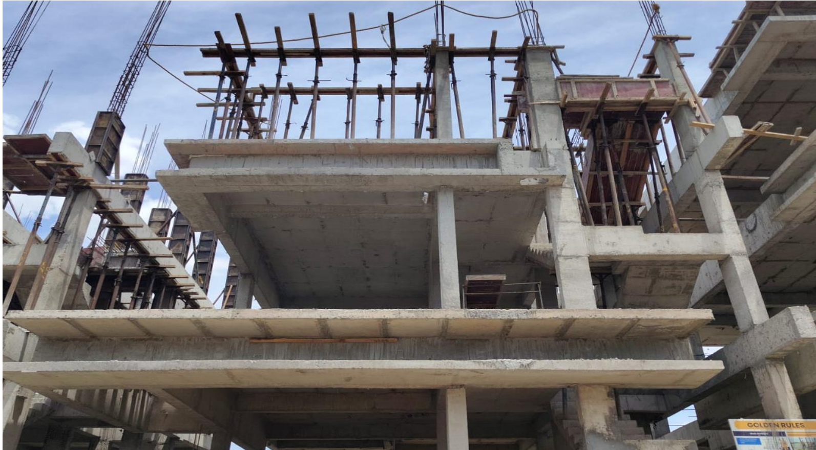
Villa No 25- SF Roof Slab Shuttering Work In Progress
