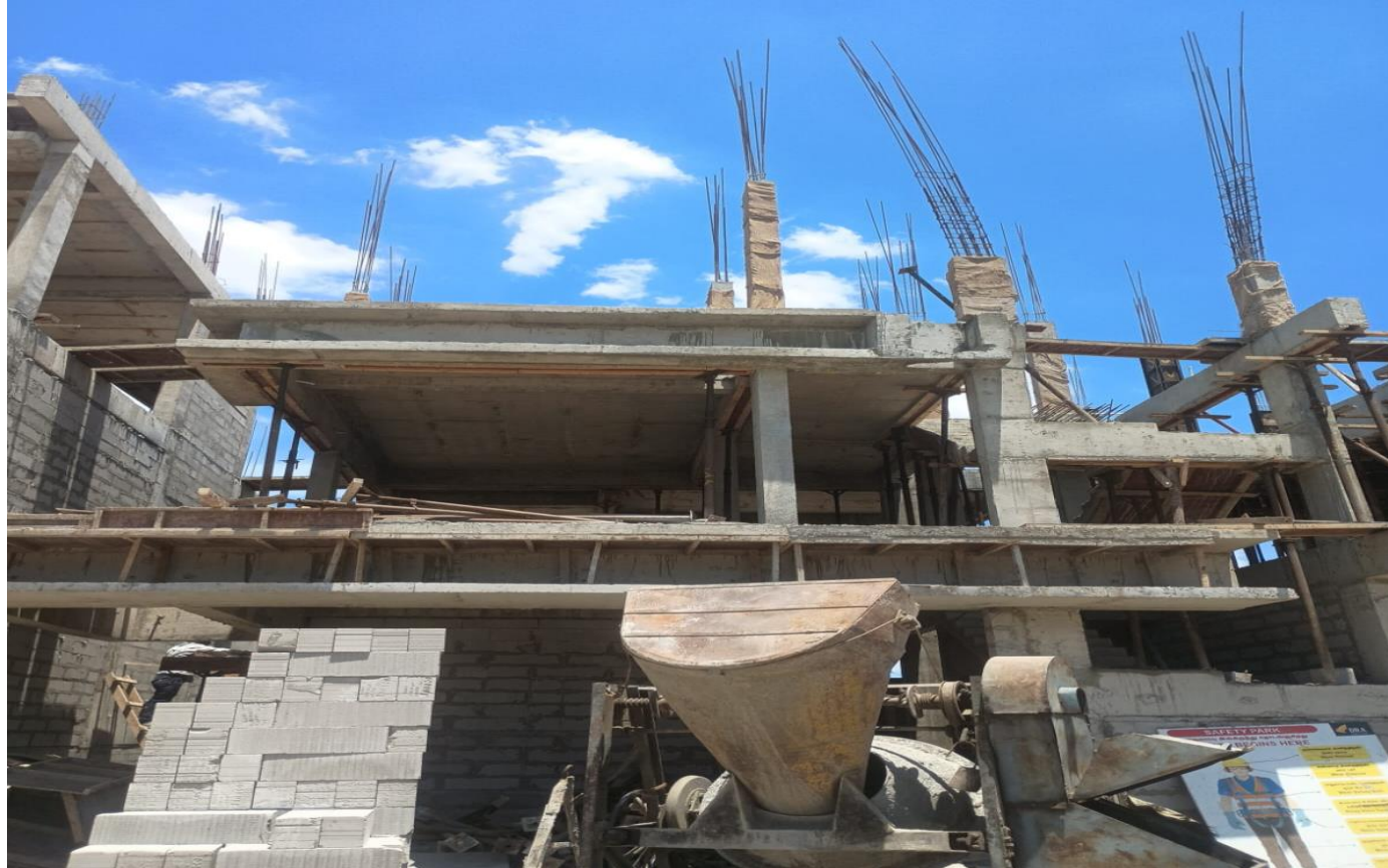
Villa No 23 –SF Column Concrete Pouring Work Completed
