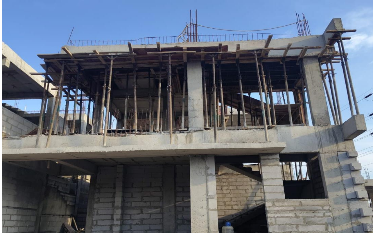
Villa No 81– FF Roof Slab Concrete Completed
