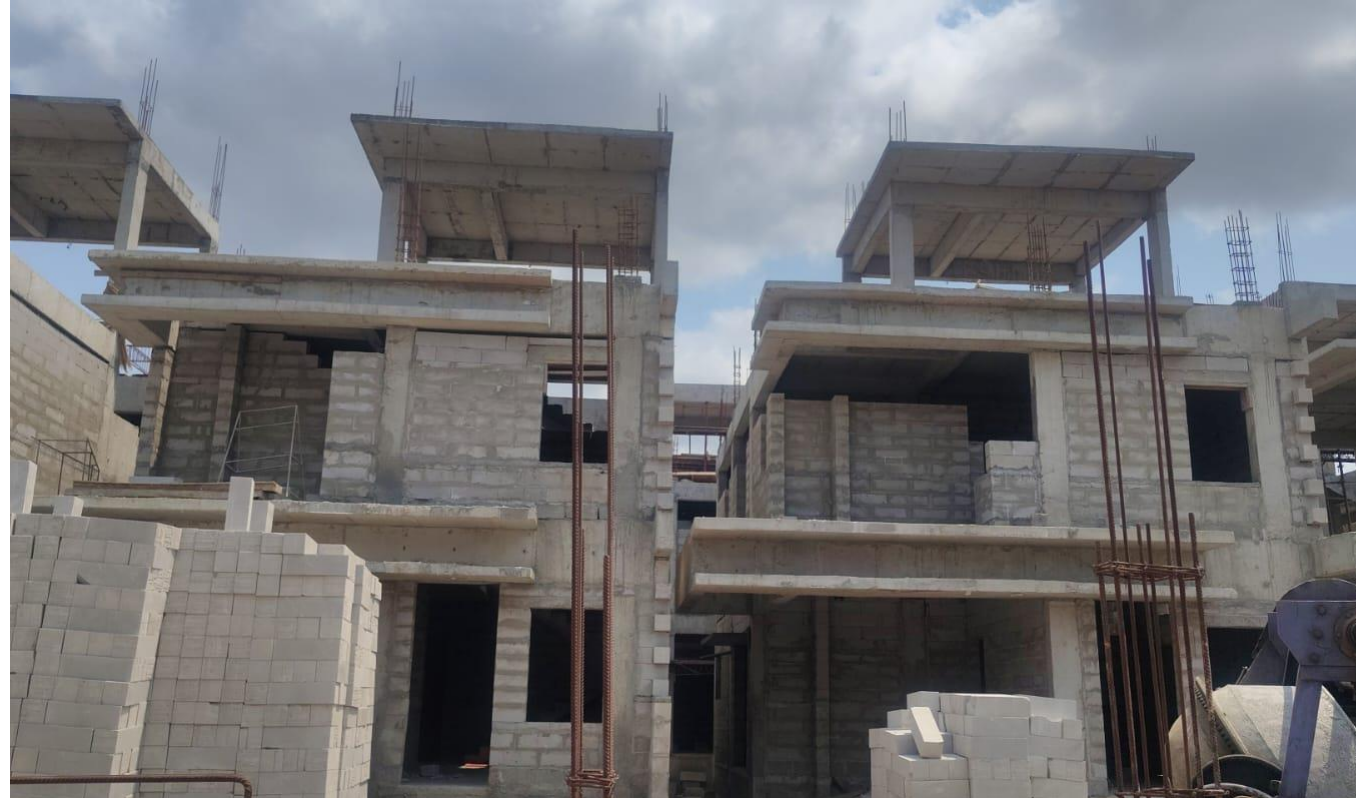
Villa No -51&52 FF Block Work In Progress
