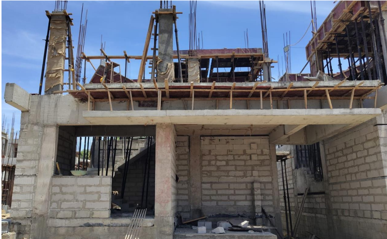
Villa No 118–FF Roof Slab Shuttering Work In Progress
