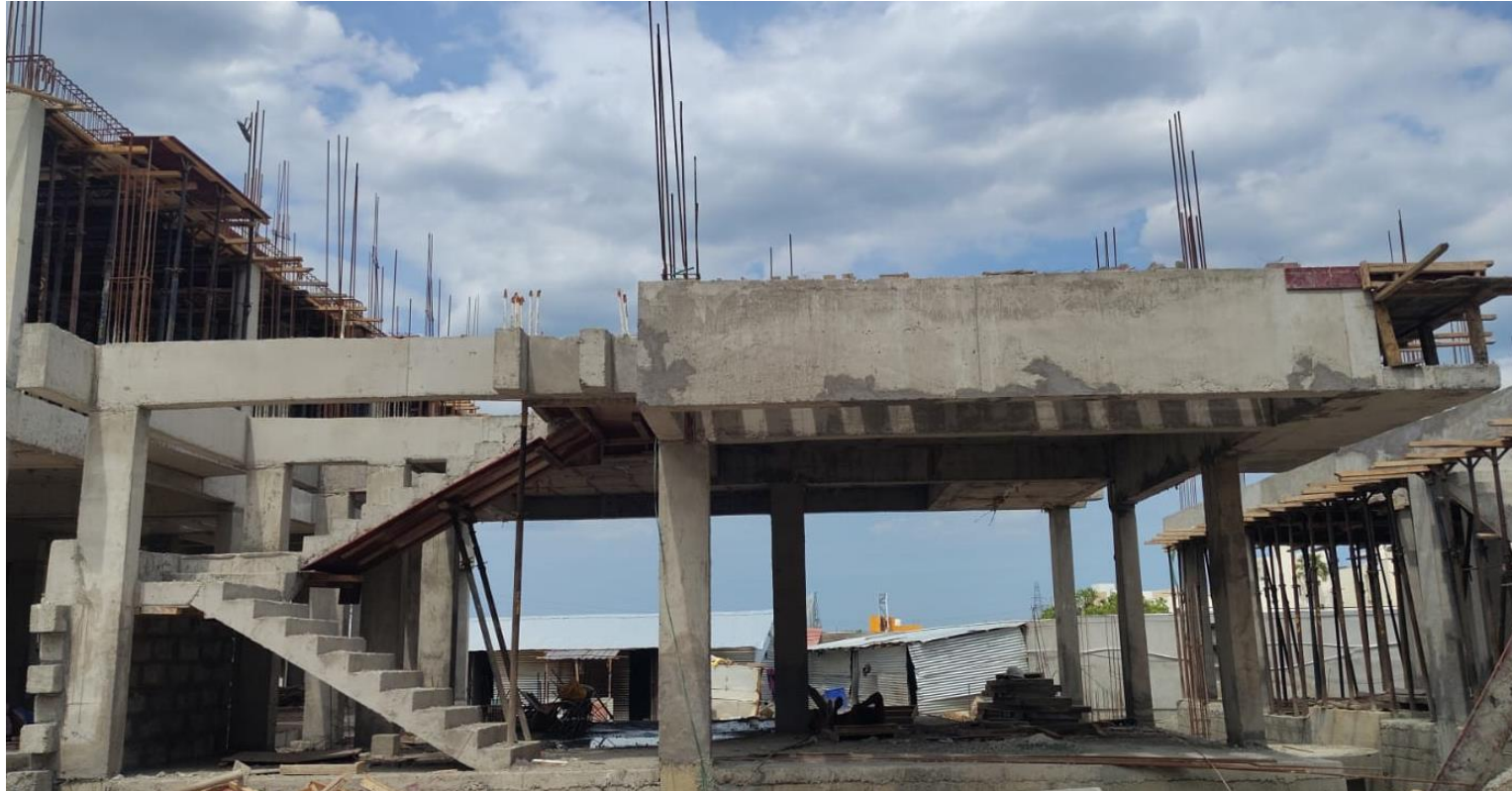
Villa No 106—GF Roof Slab Concrete Pouring Work Completed
