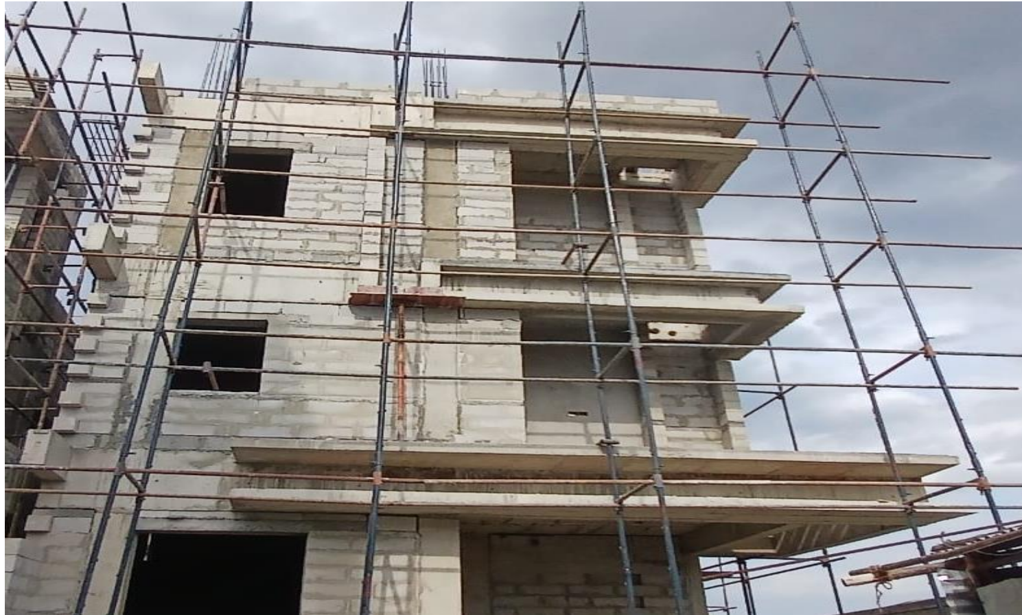
Villa No 45–External Plastering Preparation Work In Progress
