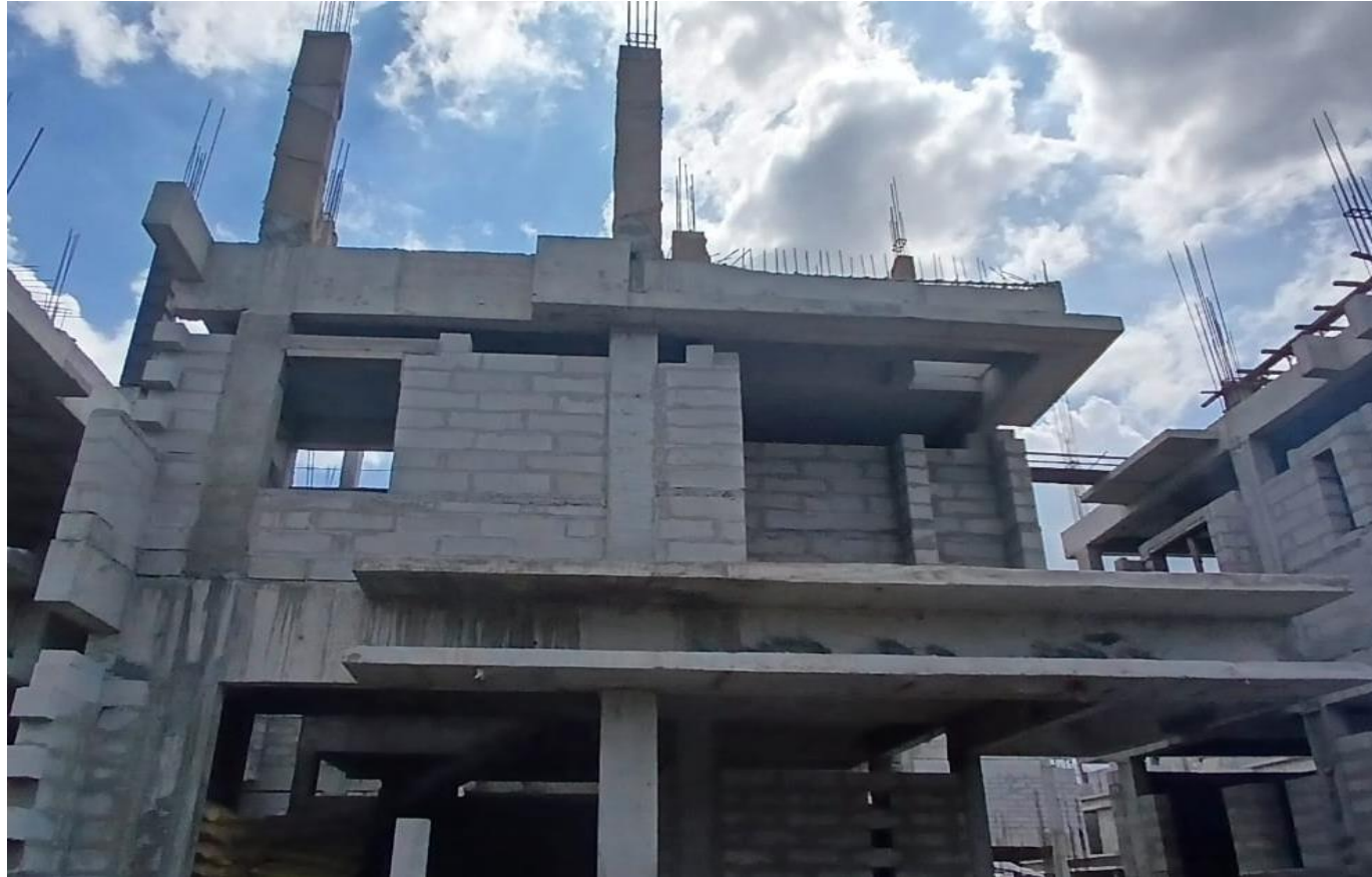
Villa No 32 –SF Column Concrete Pouring Completed'
