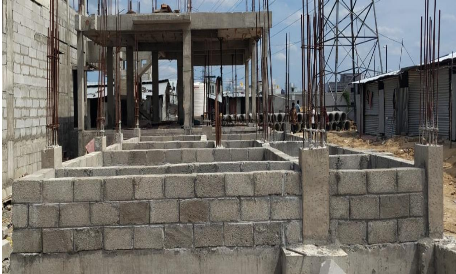
Villa No 82-Basement Block Work Completed
