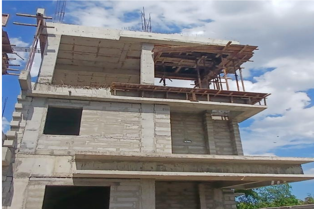
Villa No 38—FF Block Work Completed
