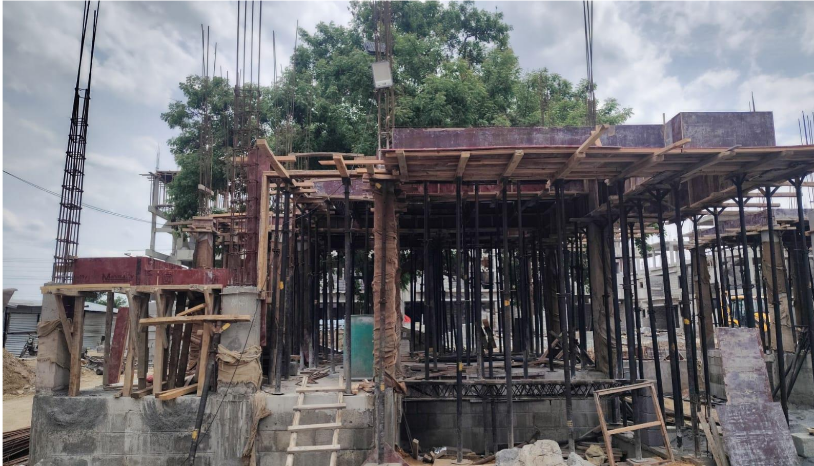
Villa No 109—GF Roof Slab Shuttering Work In Progress
