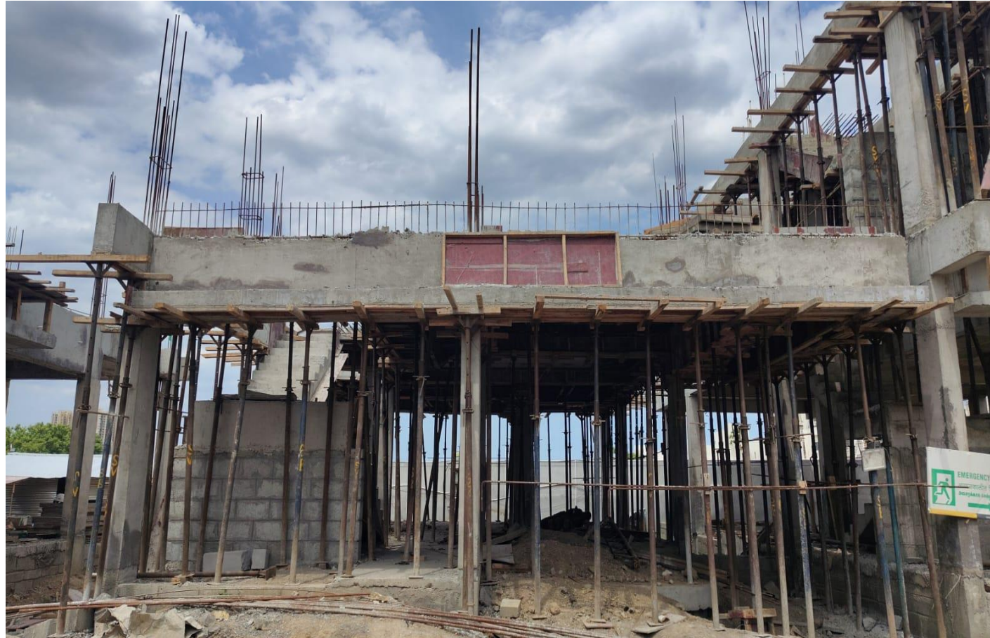
Villa No 107–GF Roof Slab Concrete Pouring Work Completed
