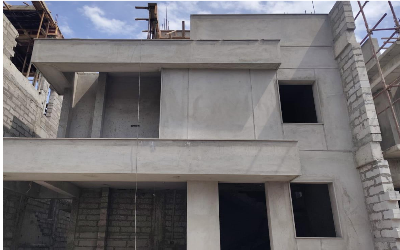
Villa No 75 –External Plastering Work In Progress
