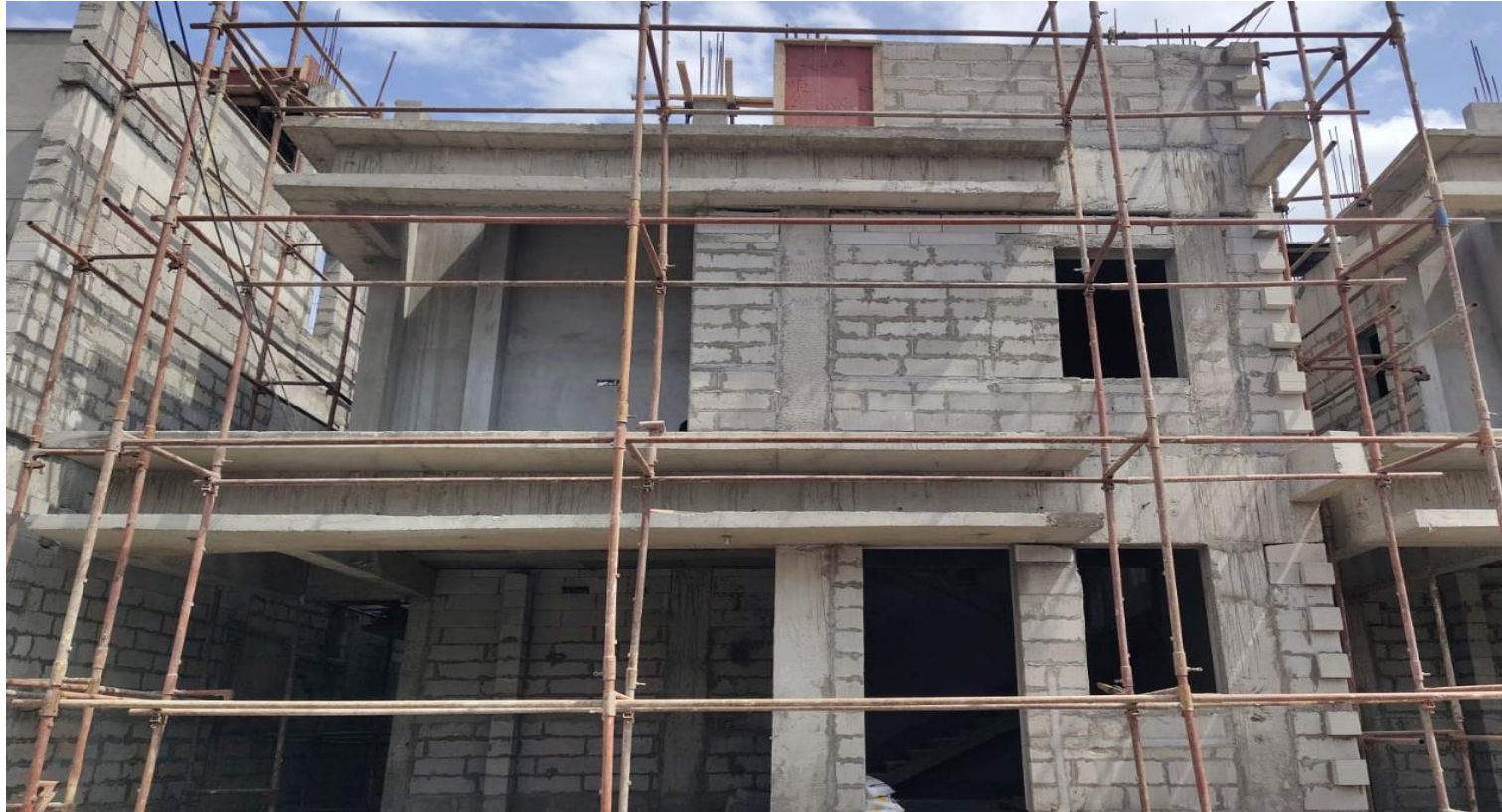
Villa No 76 –Parapet Wall Block Work In Progress
