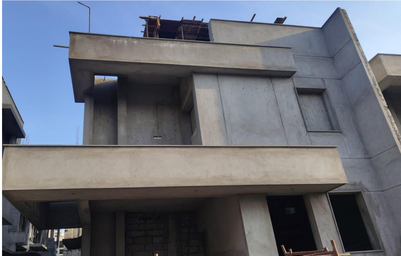
Villa No 74 –External Plastering Work In Progress
