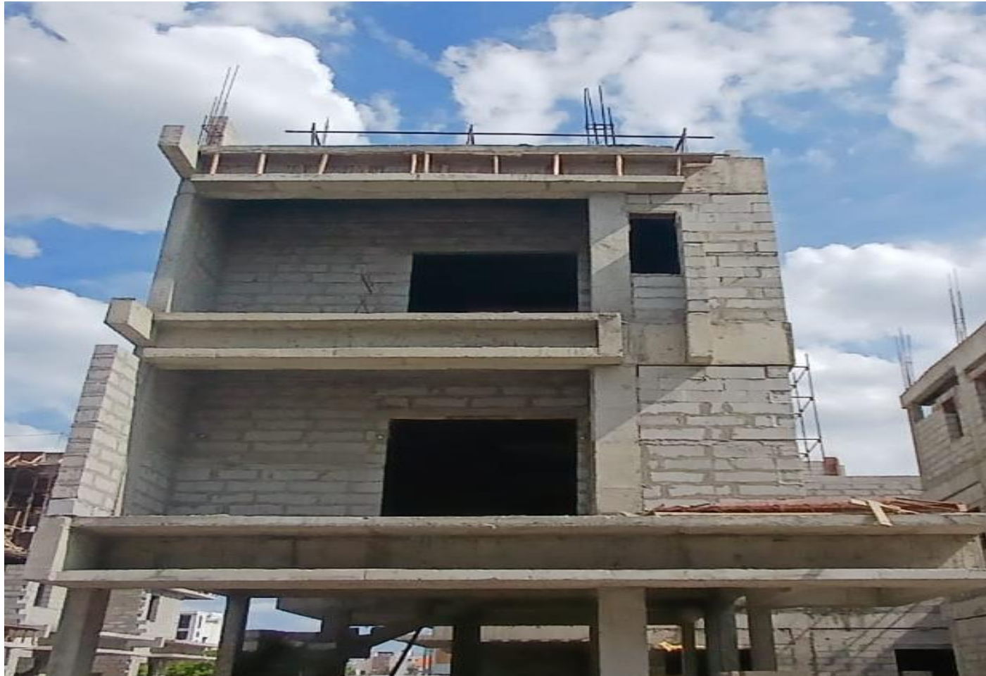
Villa No 41- Parapet Wall Block Work In Progress
