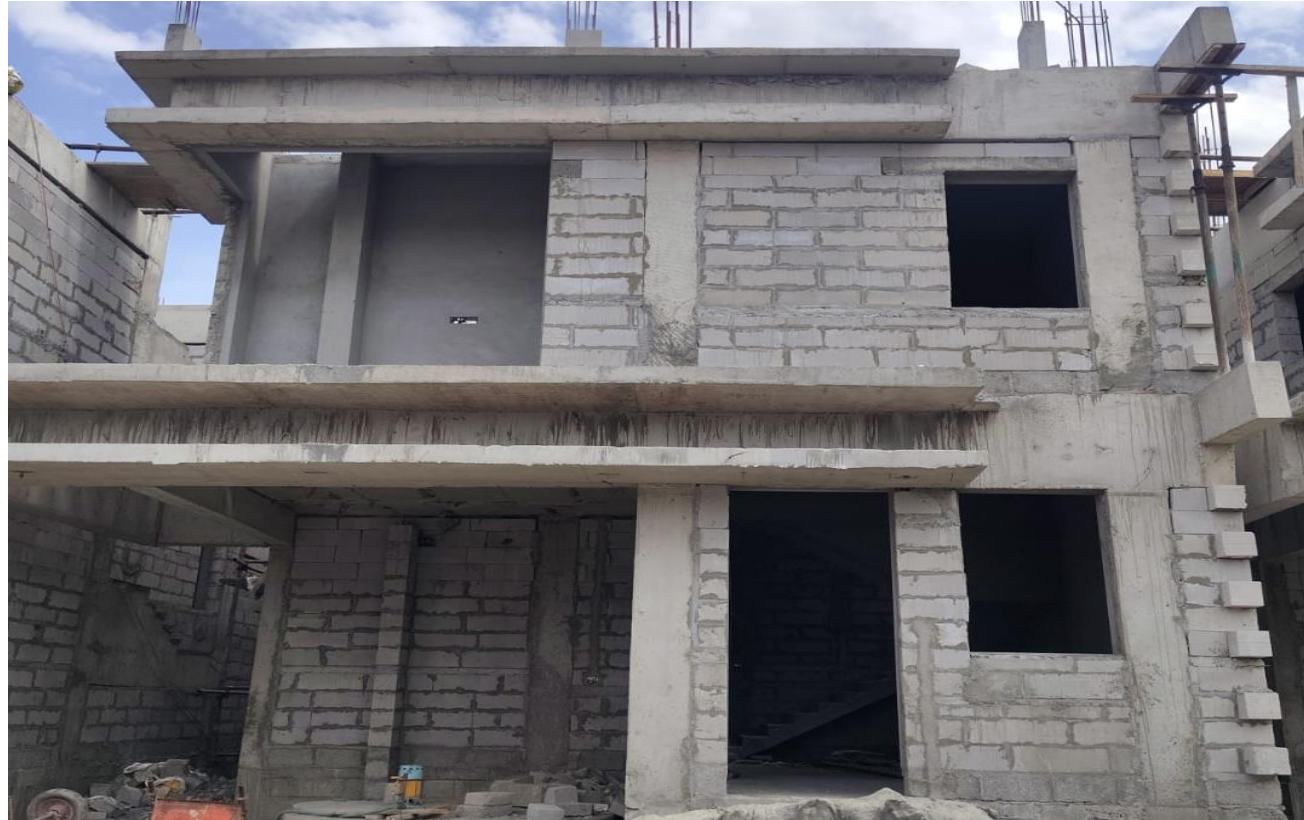
Villa No 78–FF Plastering Work In Progress
