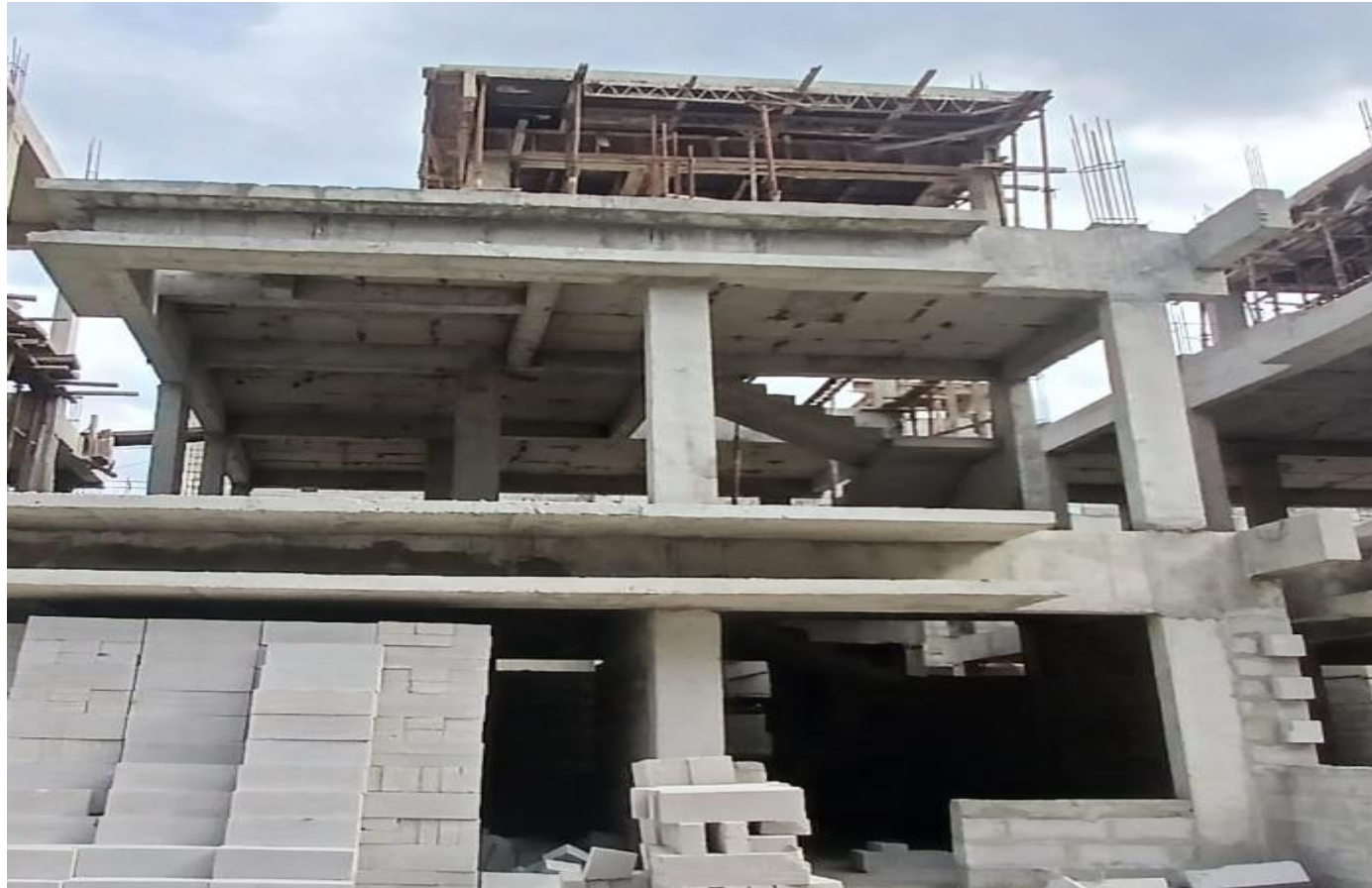
Villa No 59 –Head Room Roof Slab Concrete Pouring Completed
