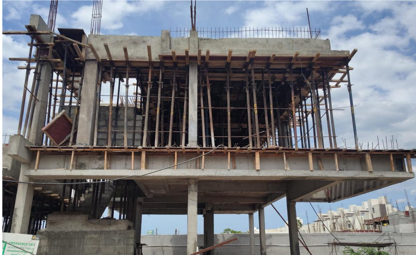
Villa No 108–FF Roof Slab Concrete Pouring Completed
