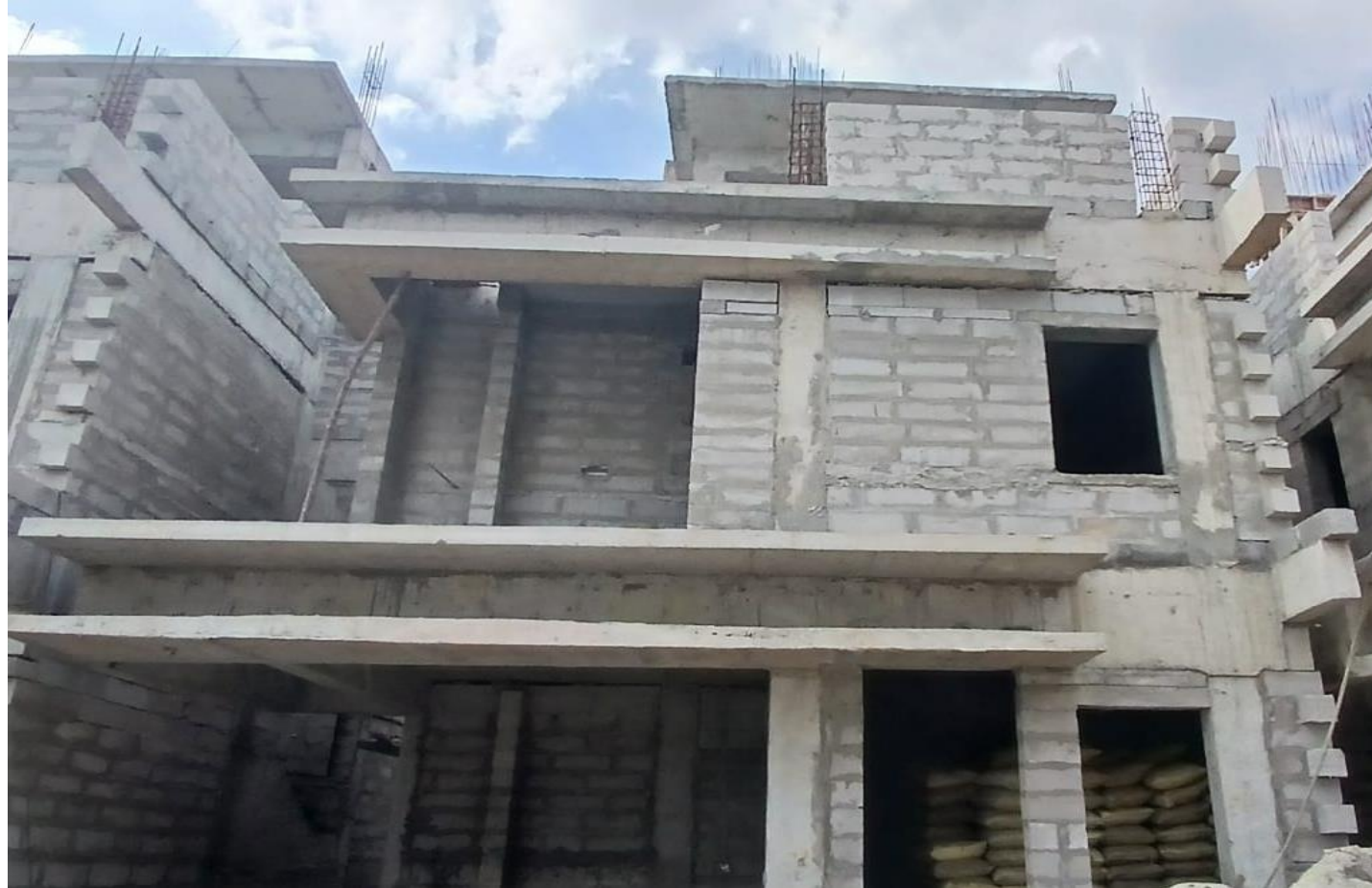
Villa No 48 –Parapet Wall Block Work In Progress
