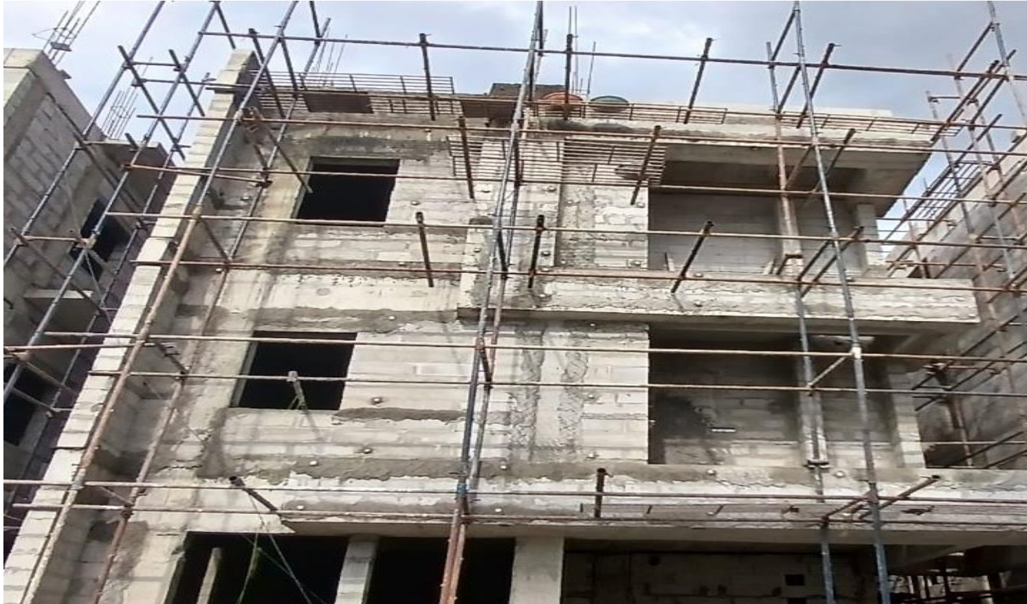
Villa No 44 –External Plastering Preparation Work In Progress
