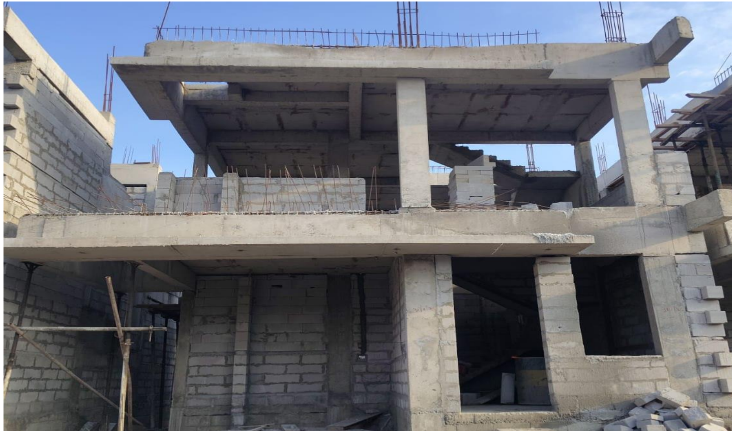
Villa No 80 –FF Block Work In Progress
