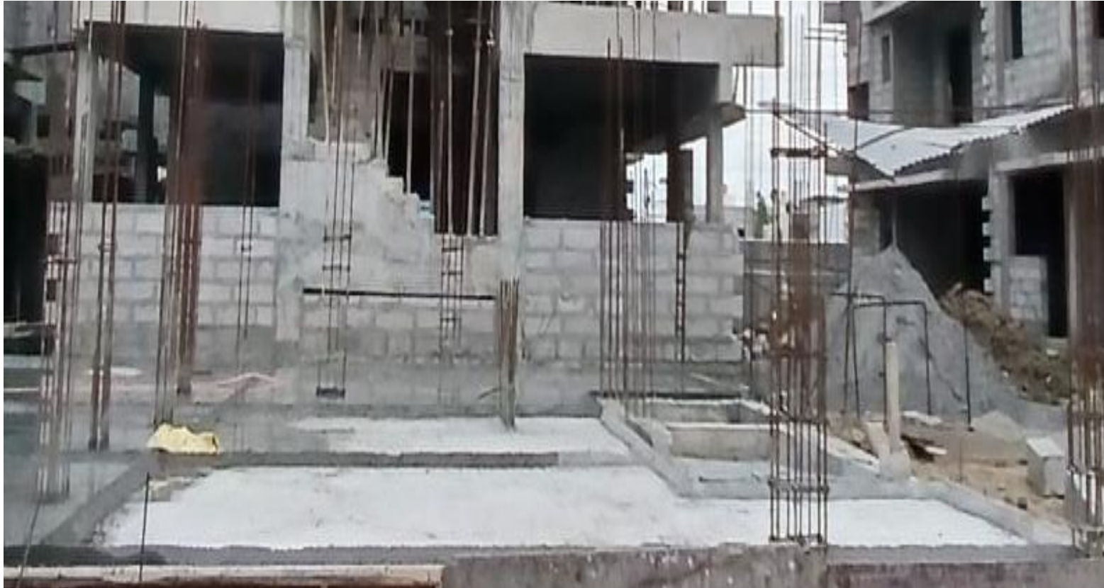
Villa No 35- GF Floor PCC Concrete Pouring work Completed
