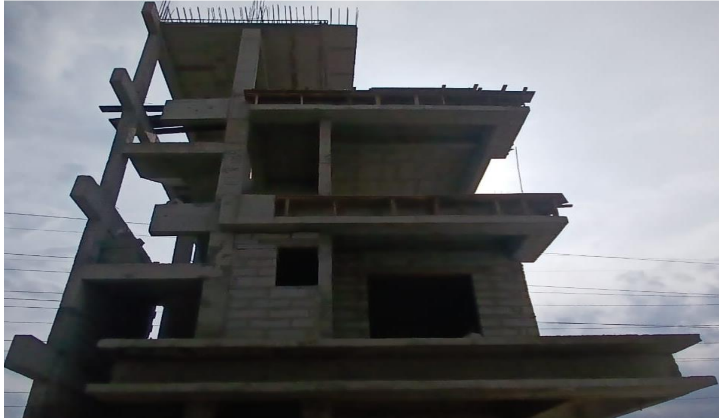
Villa No 46–SF Block Work In Progress
