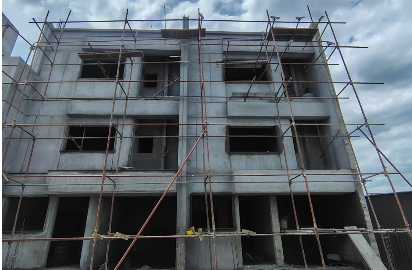
Villa No 101 to 102–External Plastering Work In Progress
