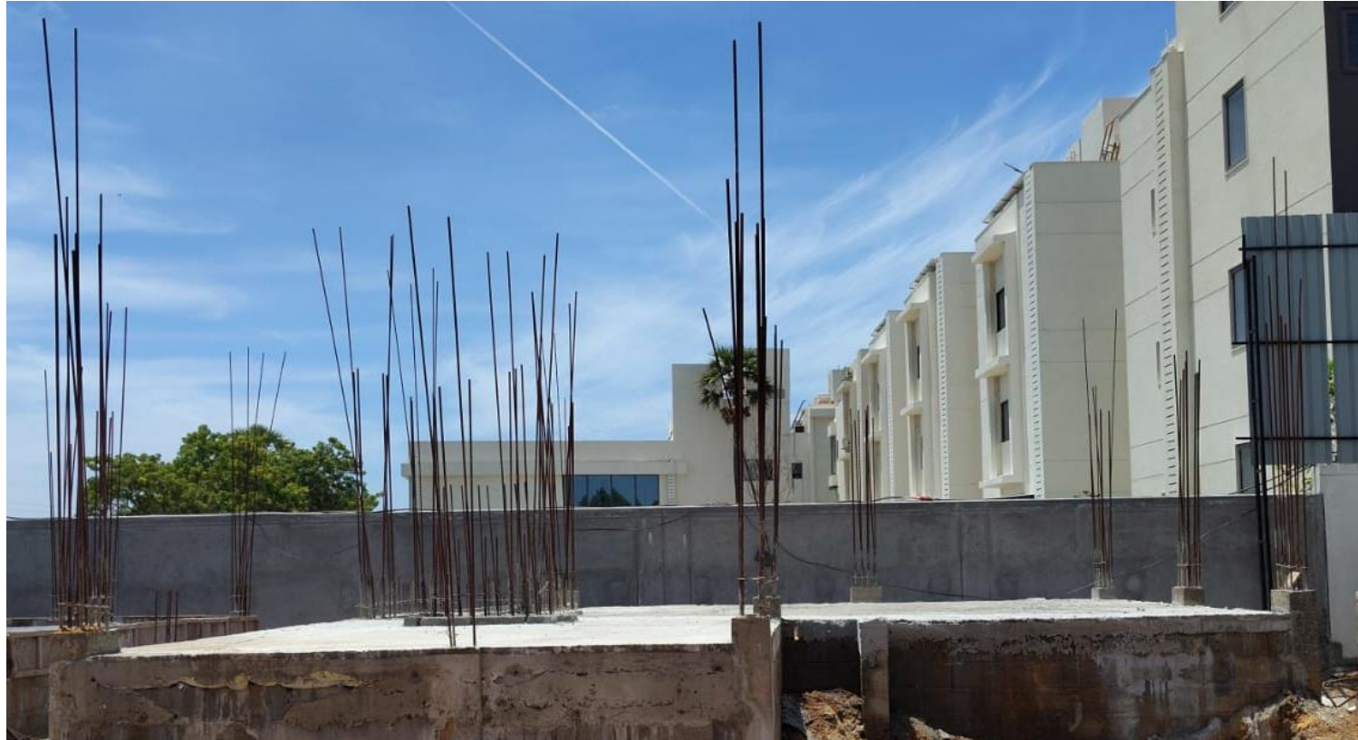
Villa No 122–GF Floor PCC Concrete Pouring Completed
