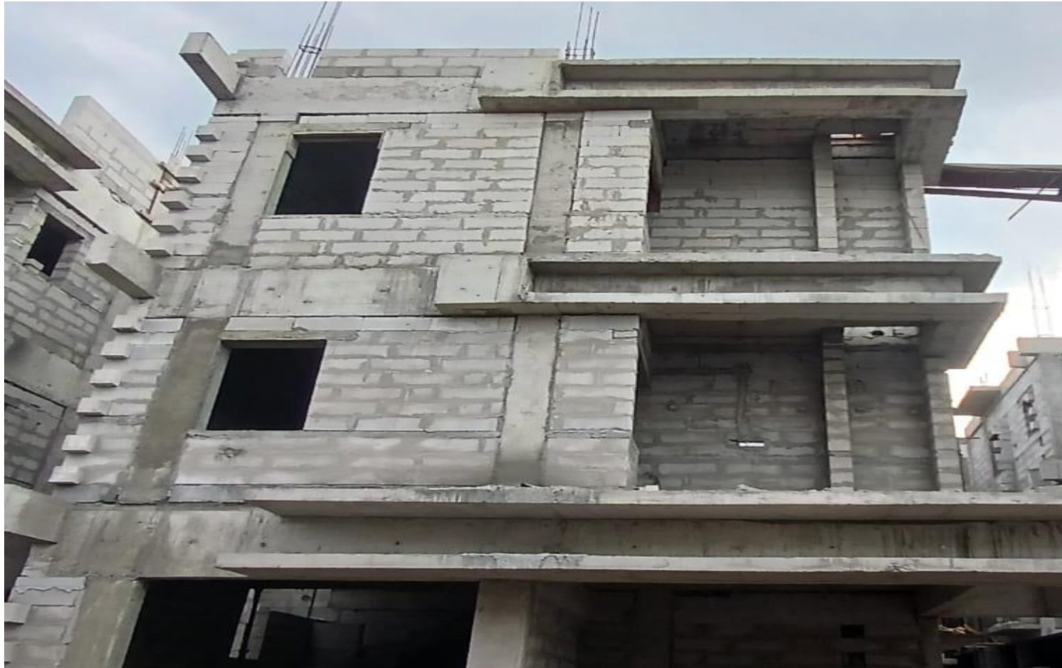
Villa No 40–Parapet Wall Block Work In Progress
