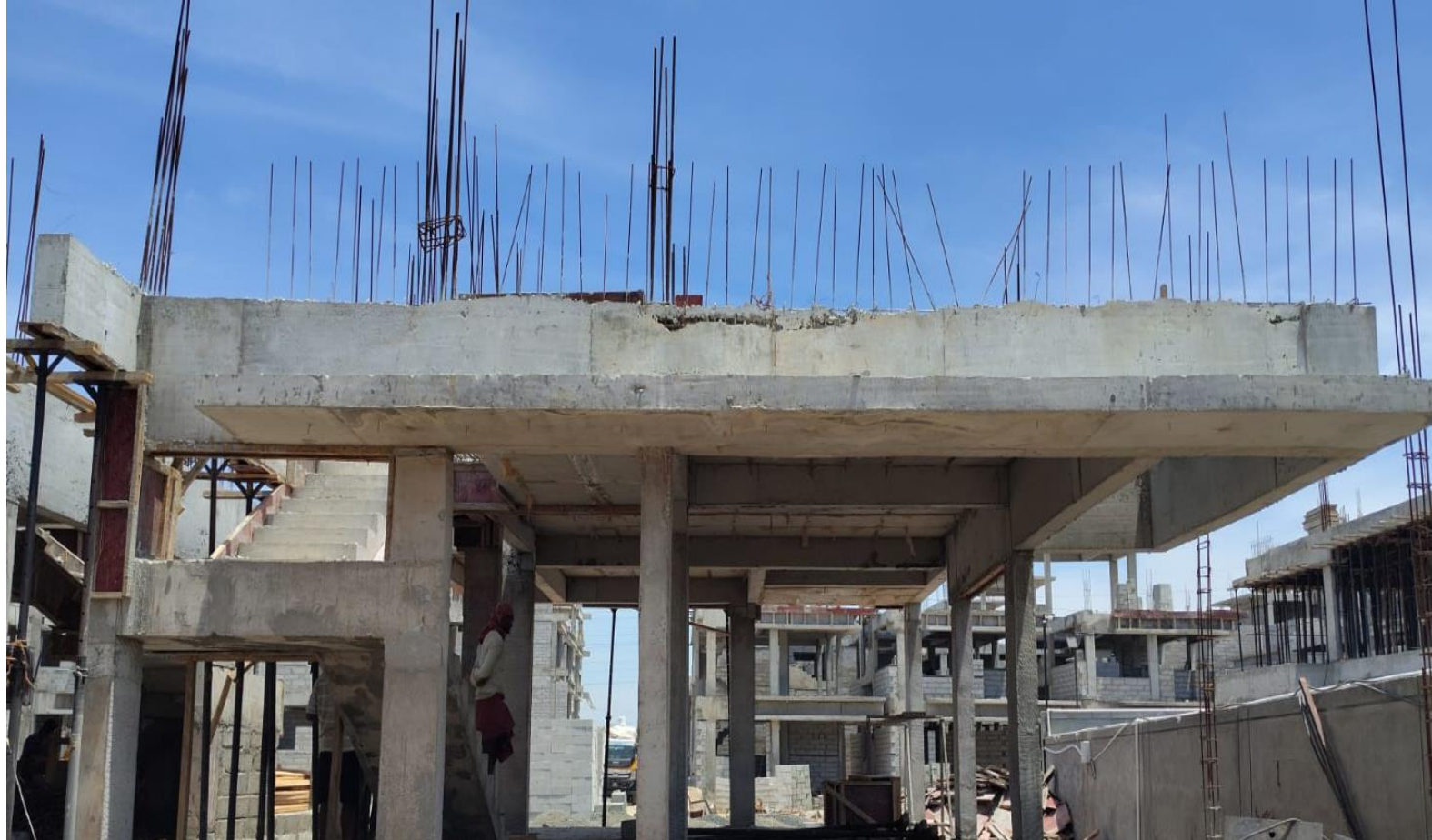
Villa No 112–GF Roof Slab Concrete Pouring Completed
