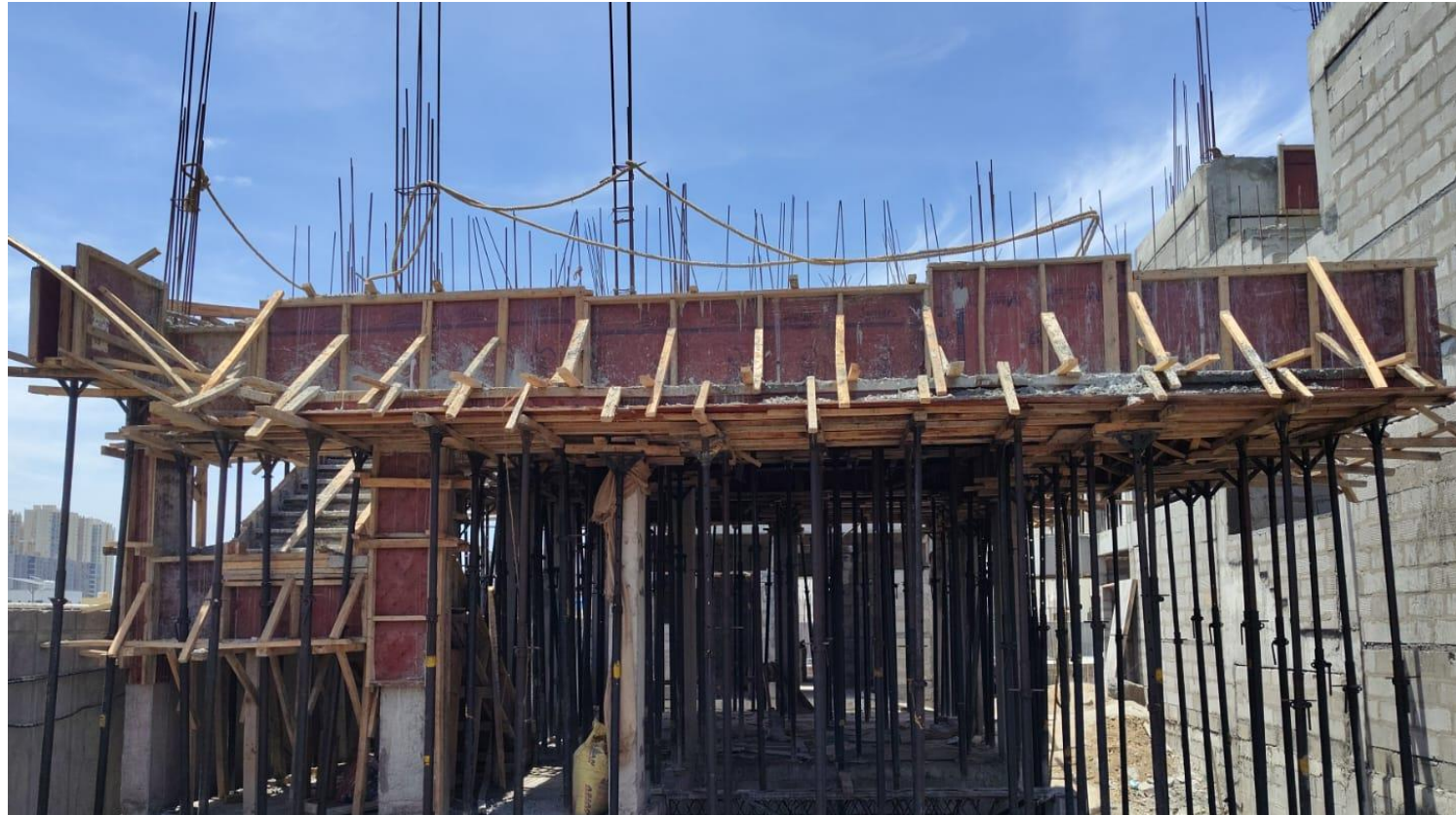
Villa No 113–GF Roof Slab Concrete Pouring Completed
