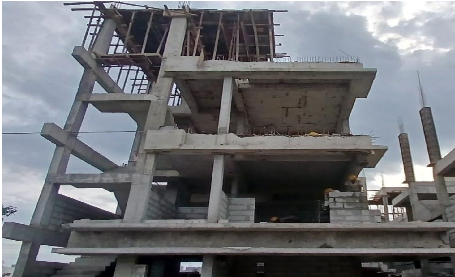
Villa No 30 –FF Block Work In Progress
