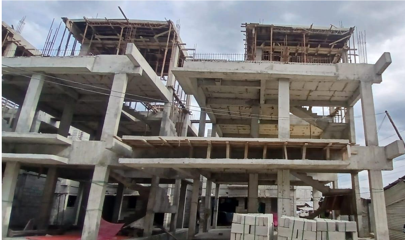
Villa No 60 & 61– Head Room Roof Slab Concrete Puring Completed
