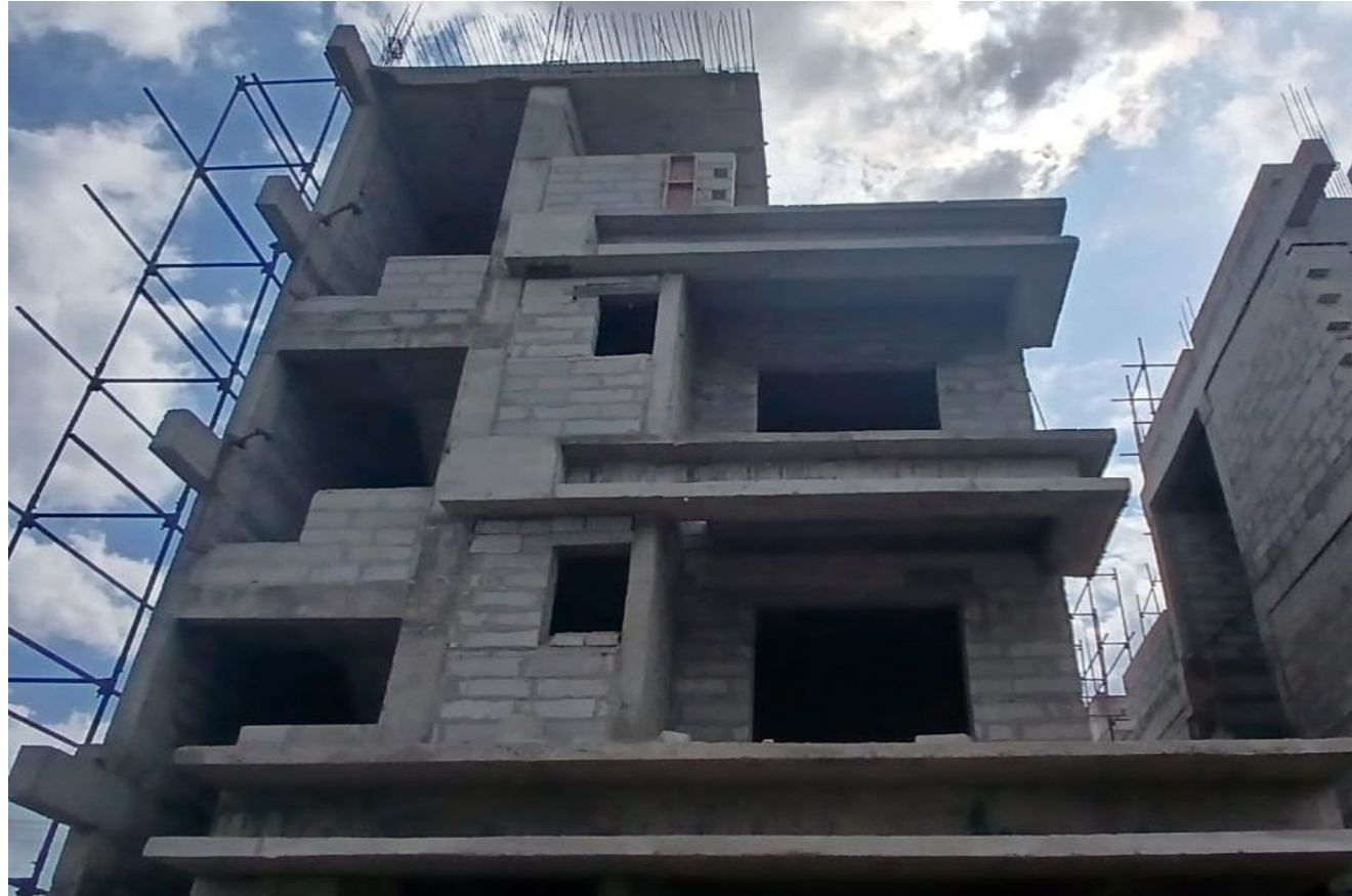
Villa No 39 –Parapet Wall Block Work In Progress
