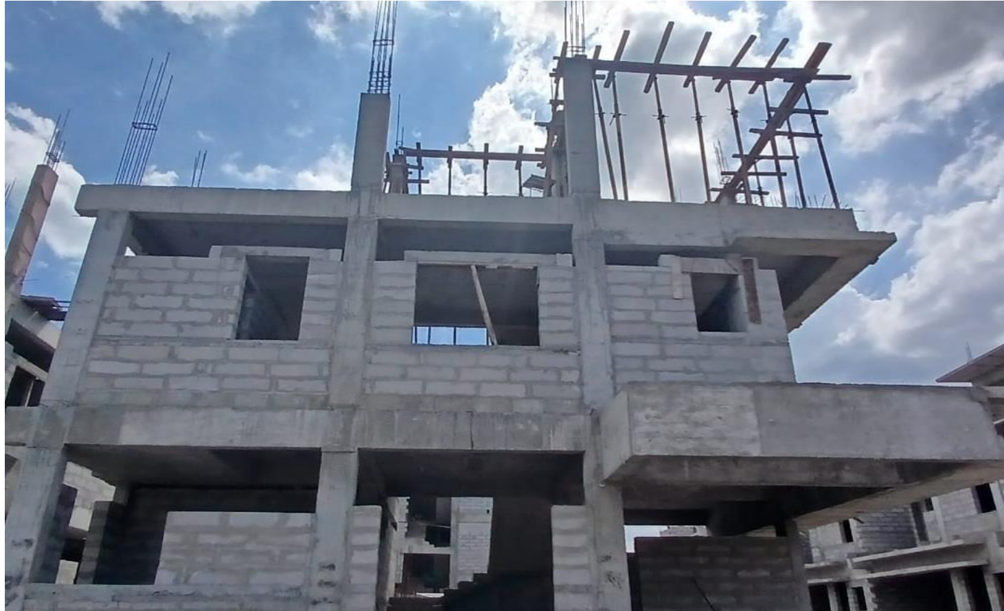
Villa No 33 –FF Block Work In Progress
