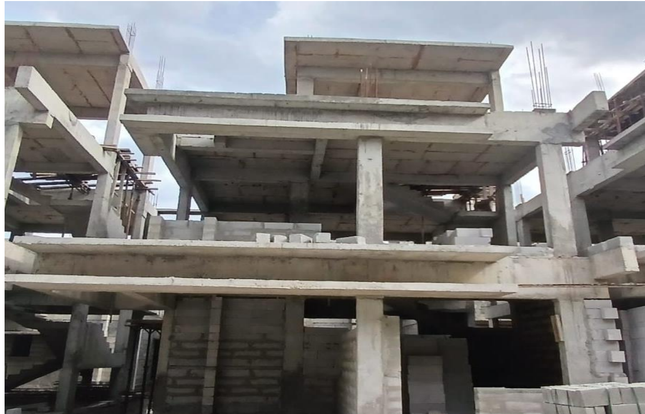
Villa No 58-FF Block Work In Progress
