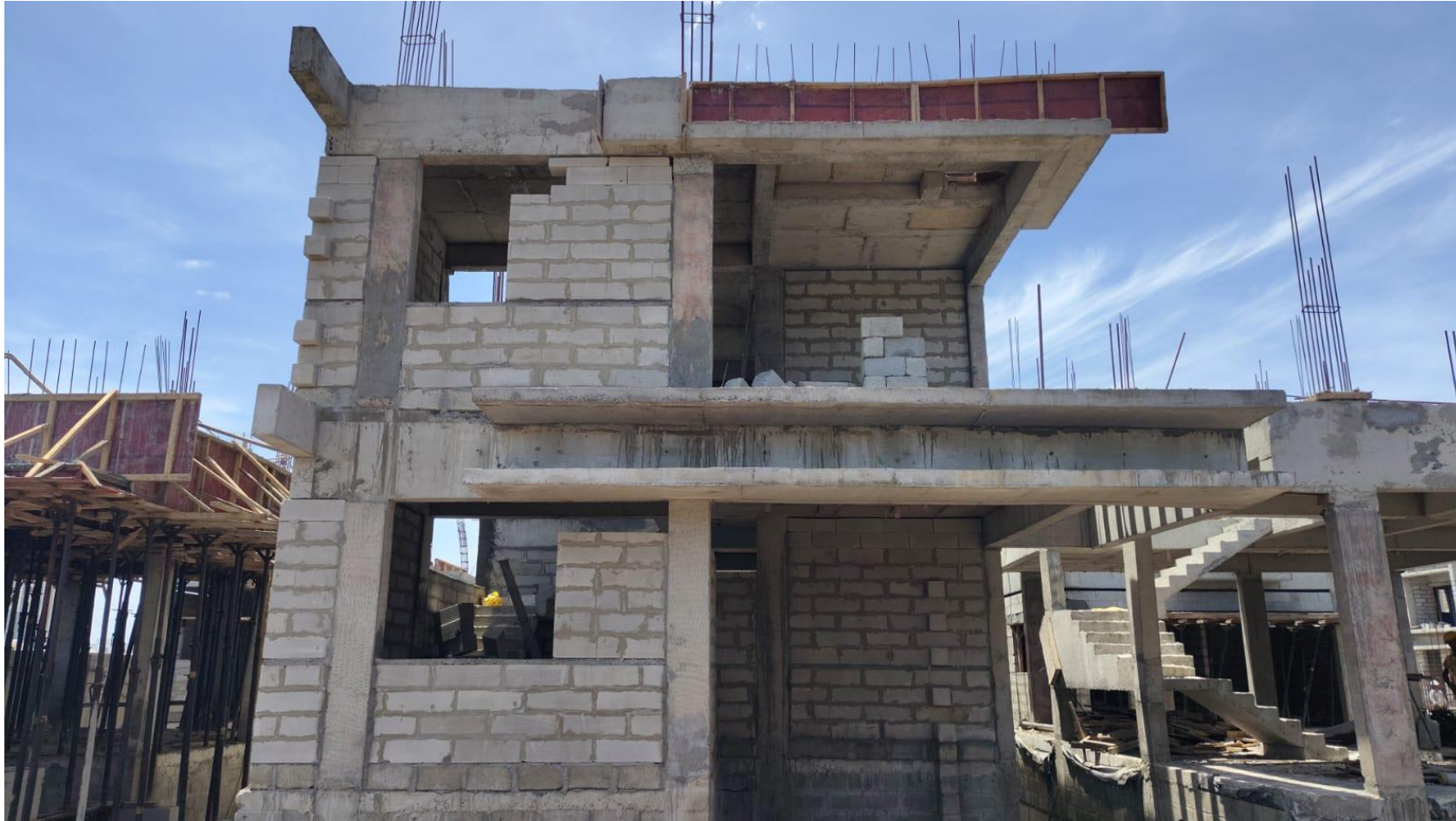
Villa No 114–FF Block Work In Progress
