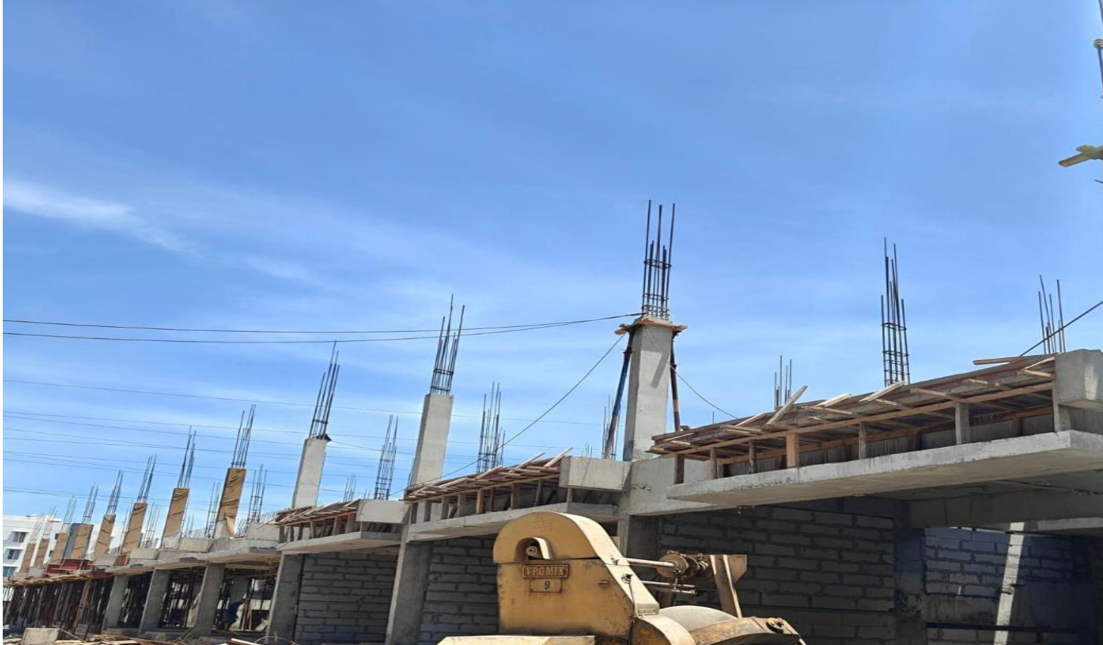
Villa No 83 to 87–FF Column Concrete Pouring Completed
