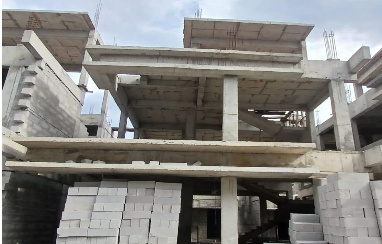
Villa No 57- Head Room Roof Slab Concrete Pouring Completed
