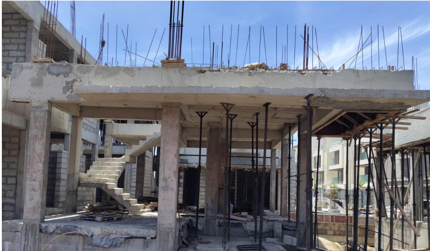
Villa No 115–GF Roof Slab Concrete Pouring Completed
