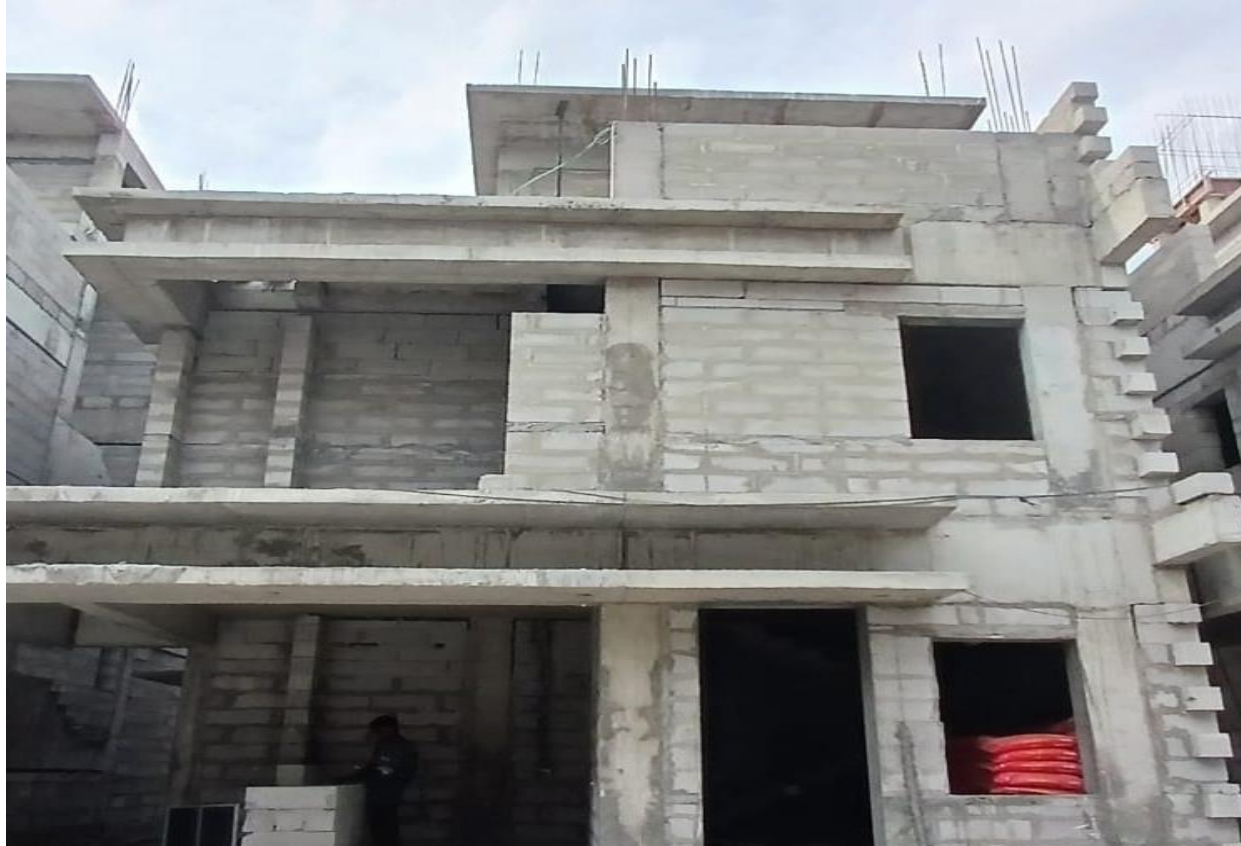
Villa No 68–Parapet Wall Block Work In Progress
