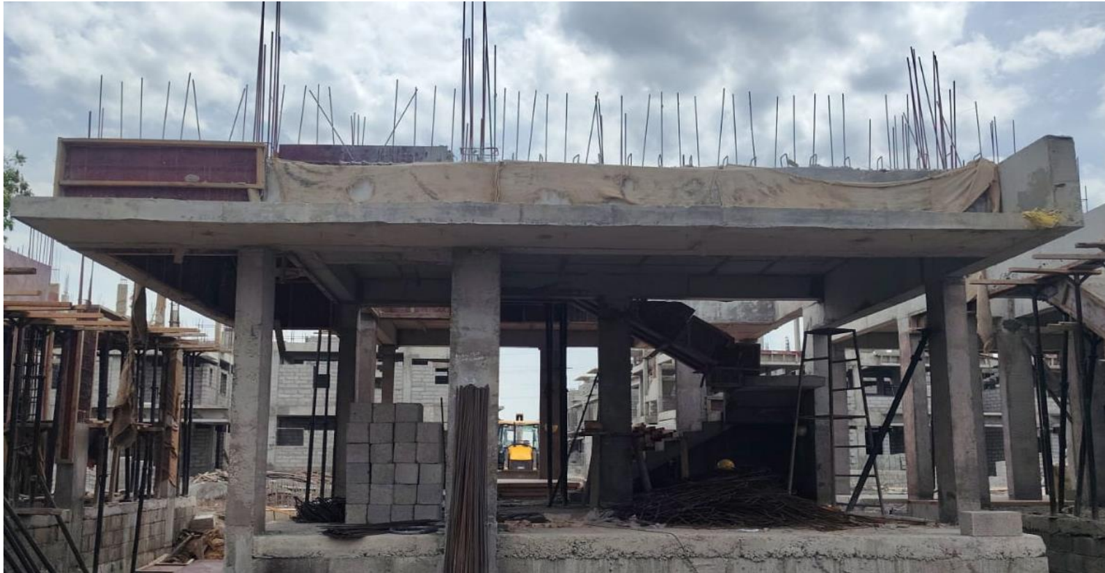
Villa No 111–GF Roof Slab Concrete Pouring Completed
