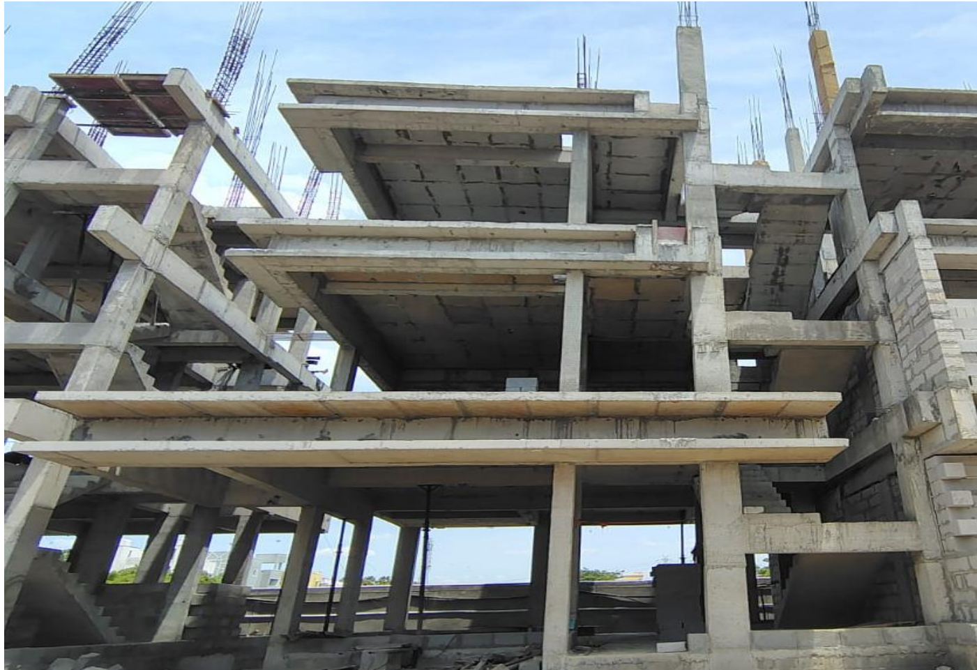
Villa No 27–Head Room Roof Slab Column Concrete Pouring Completed
