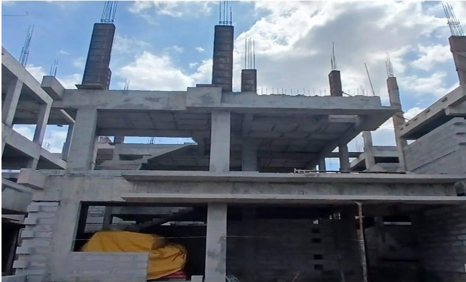
Villa No 31-SF Column Concrete Pouring Completed
