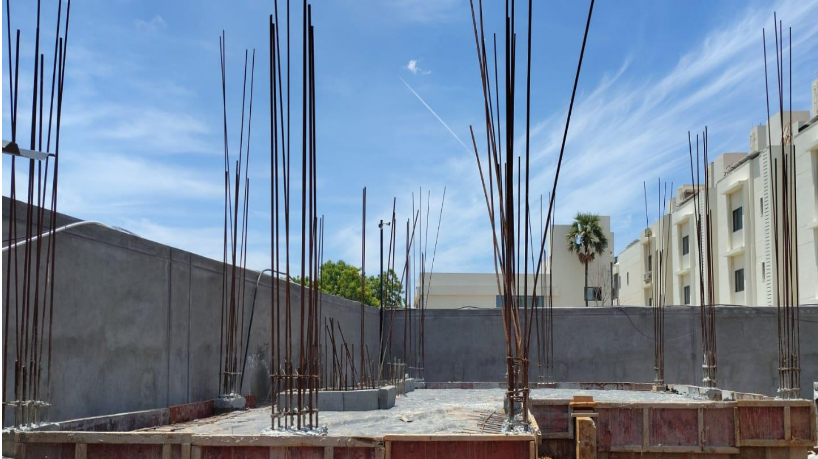
Villa No 121–GF Ready For Floor PCC
