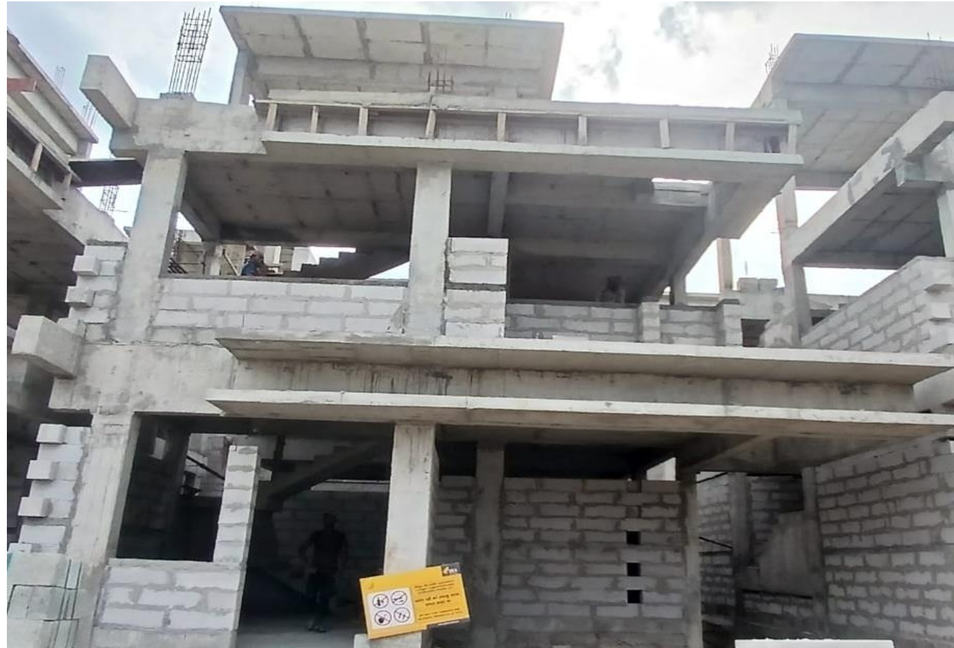
Villa No-54 GF&FF Block Work In Progress
