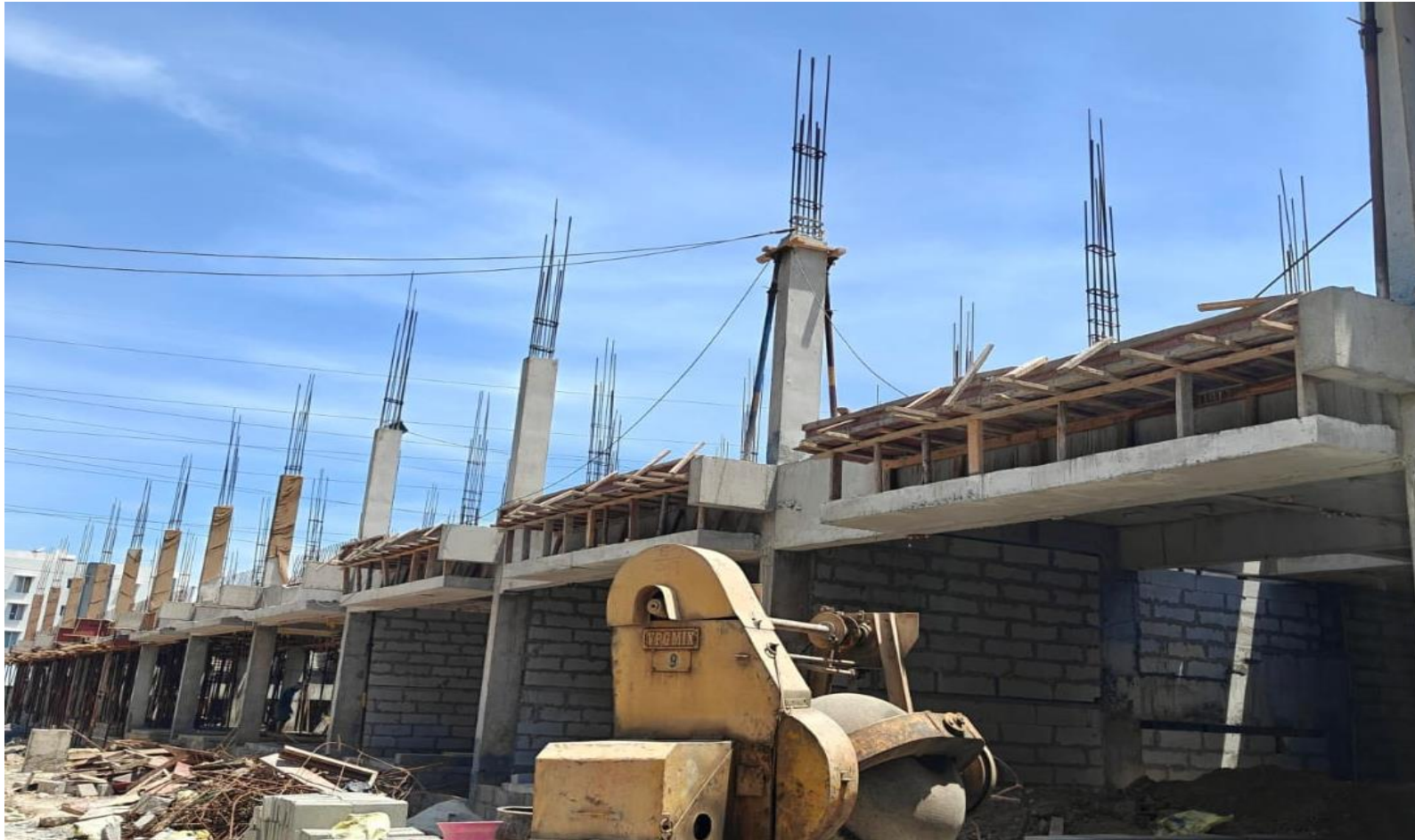
Villa No 88 To 93–FF Column Concrete Pouring Completed
