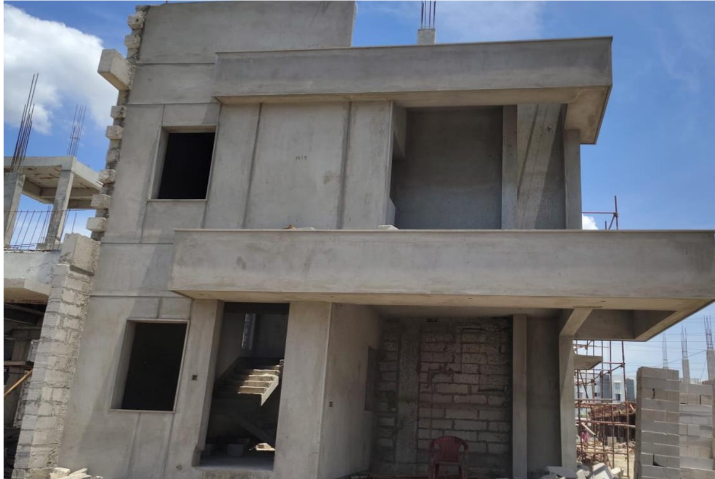
Villa No 73 –External Plastering Work In Progress
