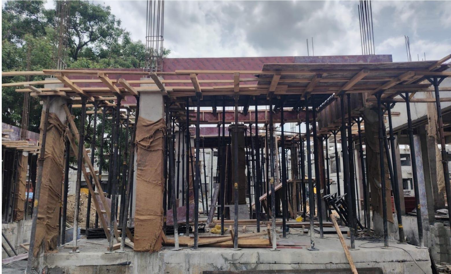
Villa No 110—GF Roof Slab Shuttering Work In Progress
