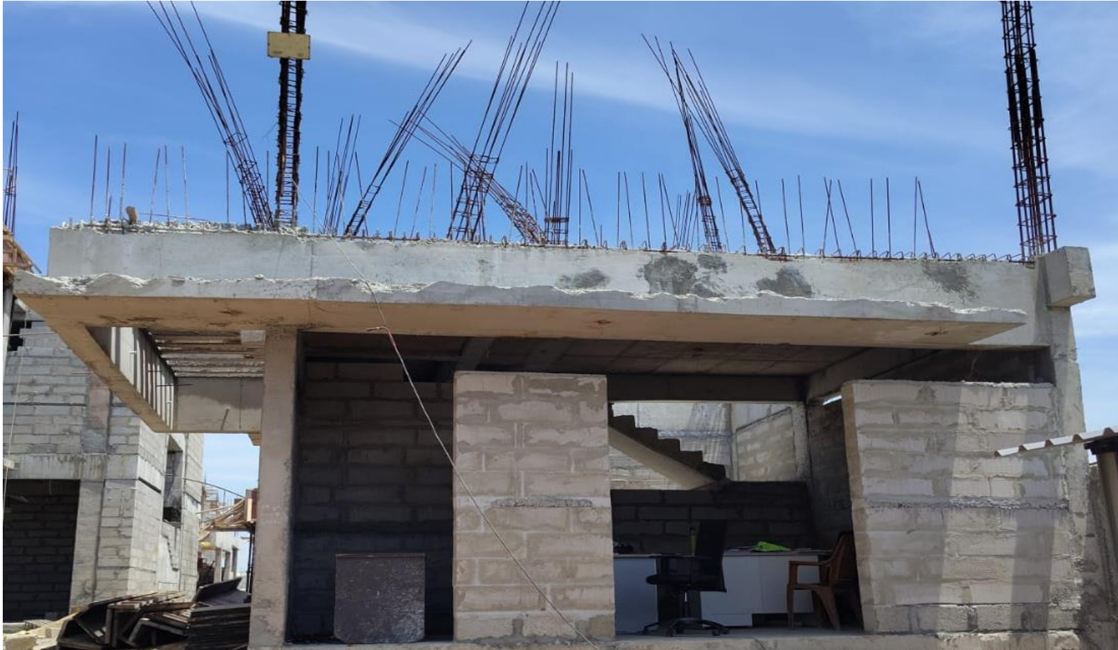
Villa No 120–FF Column Reinforcement Work In Progress
