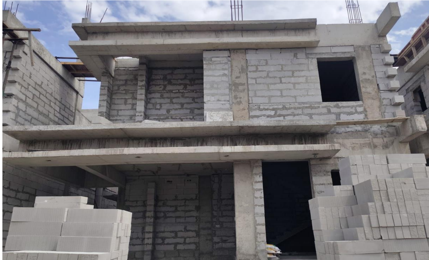
Villa No 79 –Parapet Wall Block Work In Progress
