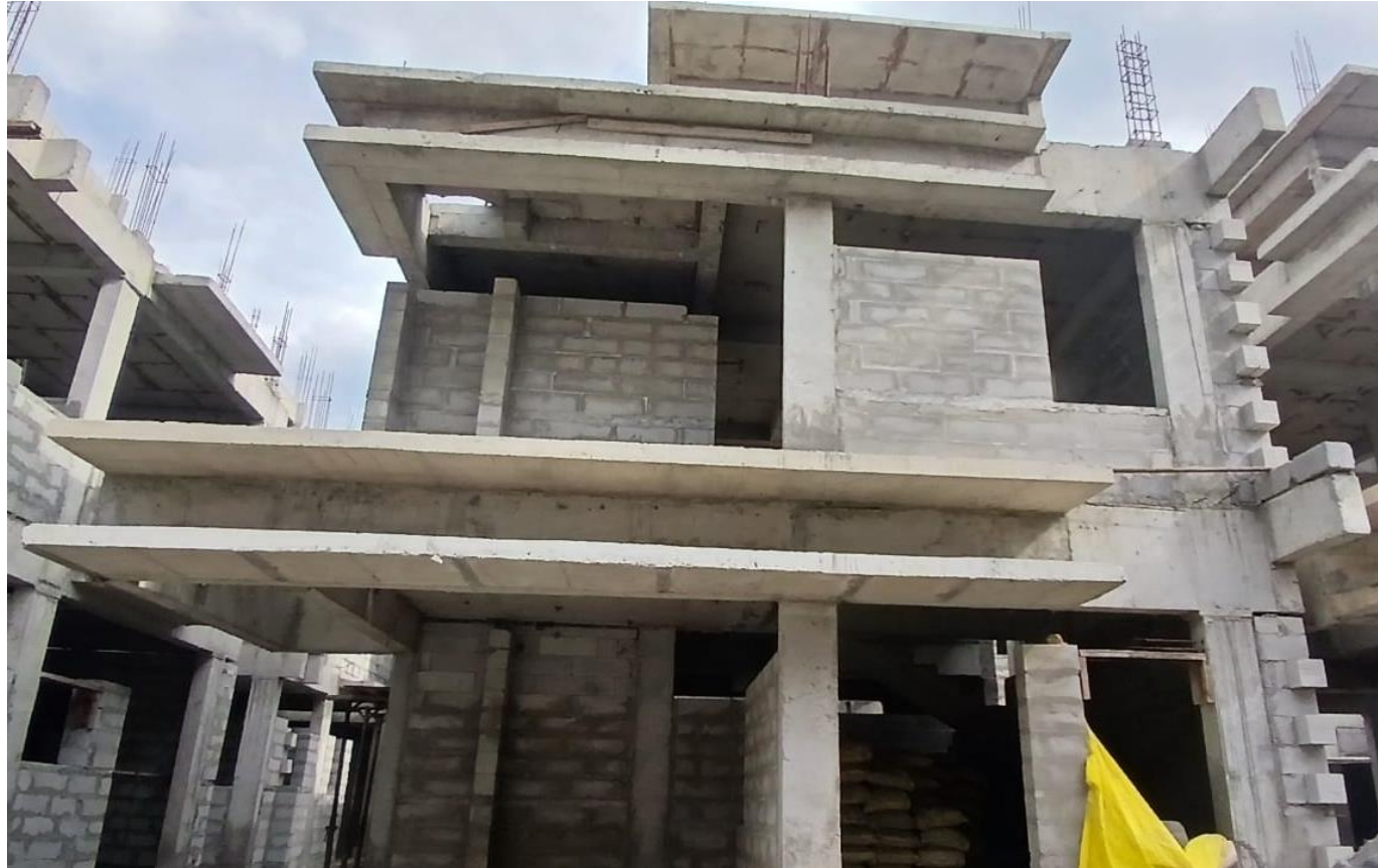
Villa No 56 – FF Block Work In Progress
