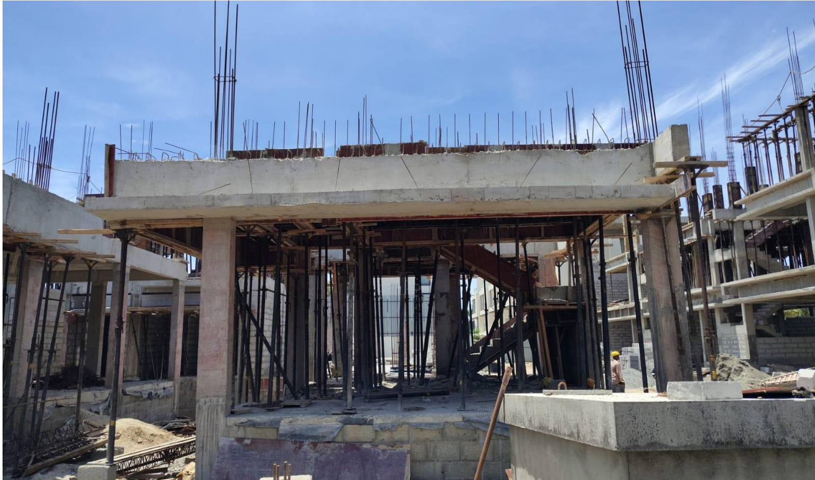
Villa No 116–GF Roof Slab Concrete Pouring Work Completed
