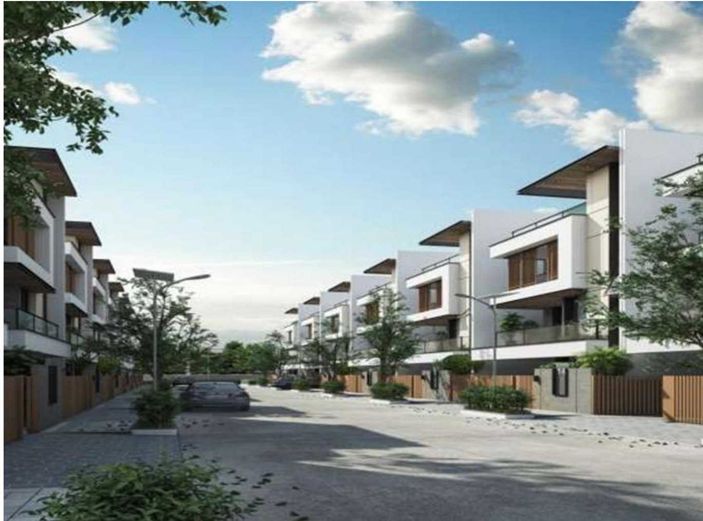
DRA INARA Monthly Progress Photos –June 2026– Phase 3 (Row Villas)
