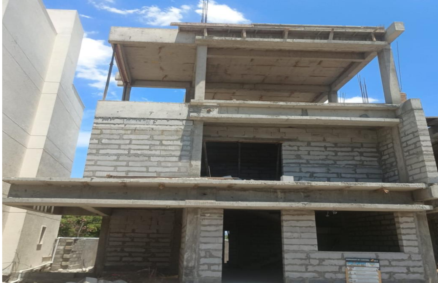
Villa No 22 –FF Block work Completed
