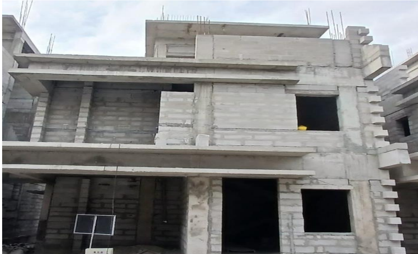
Villa No 69–Parapet Wall Block Work In Progress
