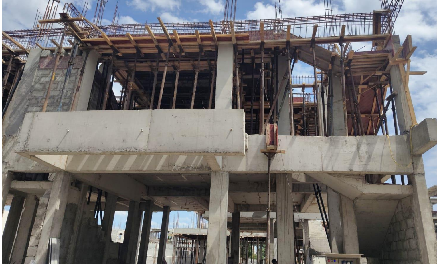
Villa No 105 – FF Roof Slab Reinforcement Work In Progress
