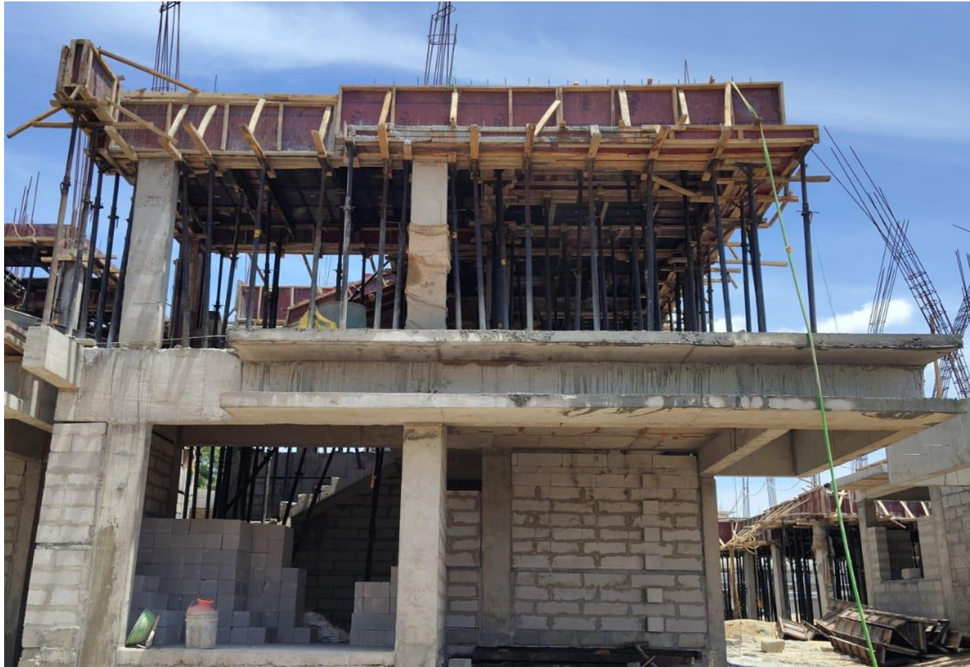
Villa No 119–FF Roof Slab Concrete Pouring Completed
