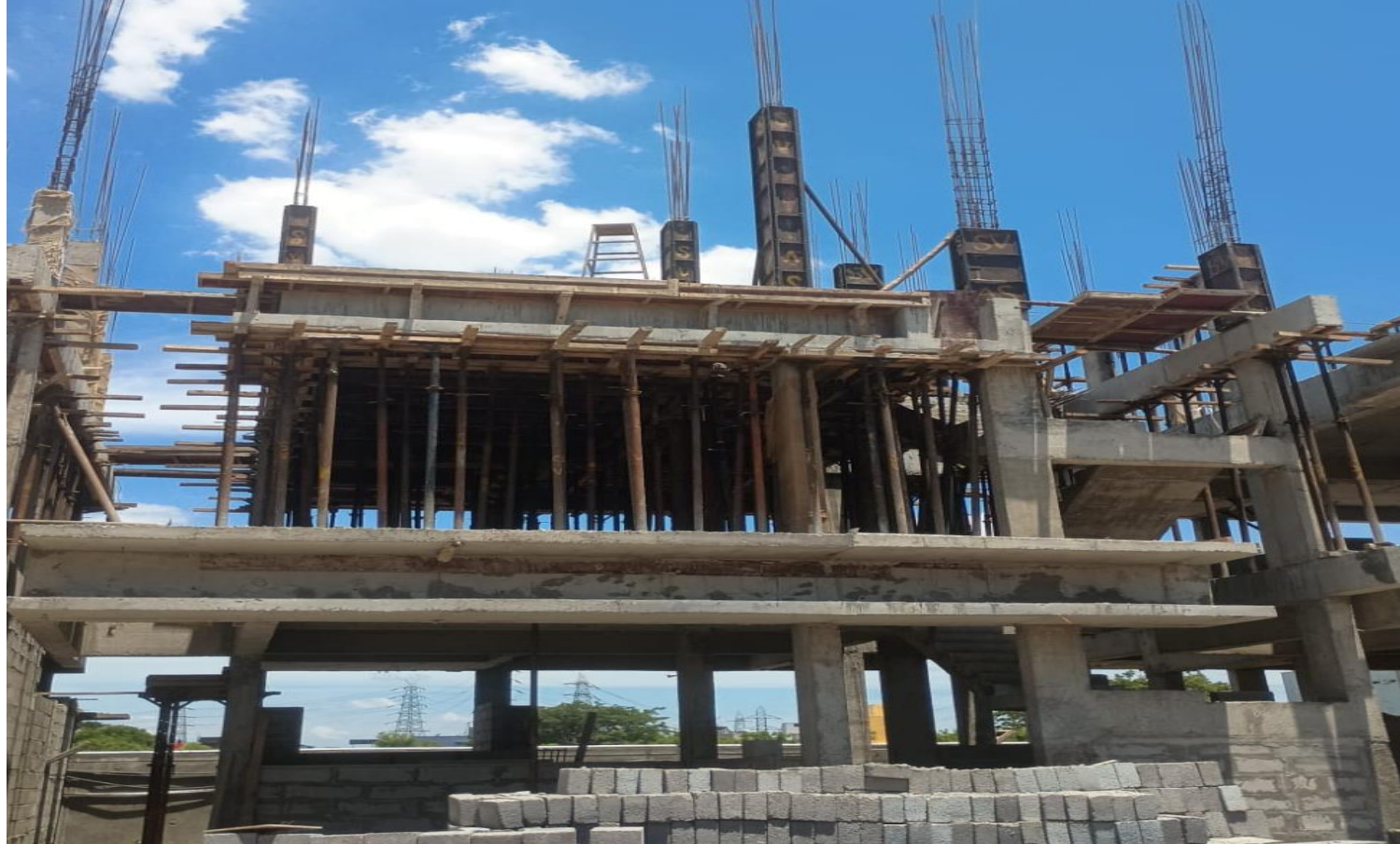
Villa No 24- SF Column Concrete Pouring Work Completed
