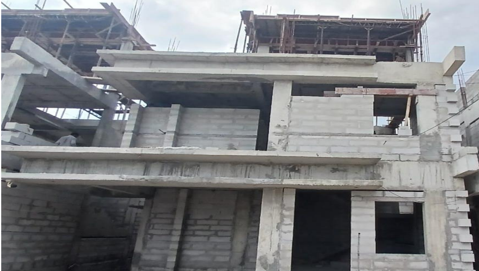
Villa No-64 FF Block Work In Progress
