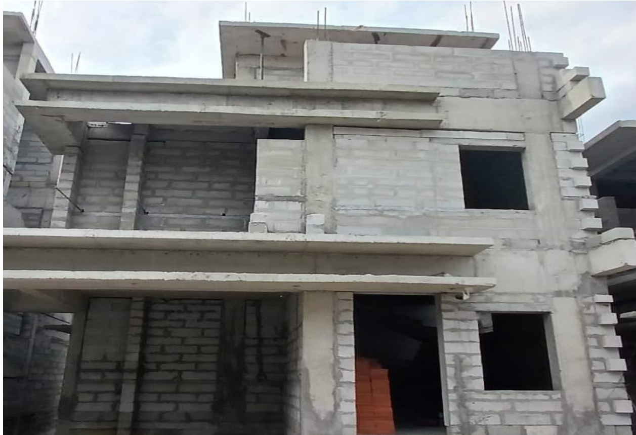
Villa No 70 – Parapet Wall Block Work In Progress
