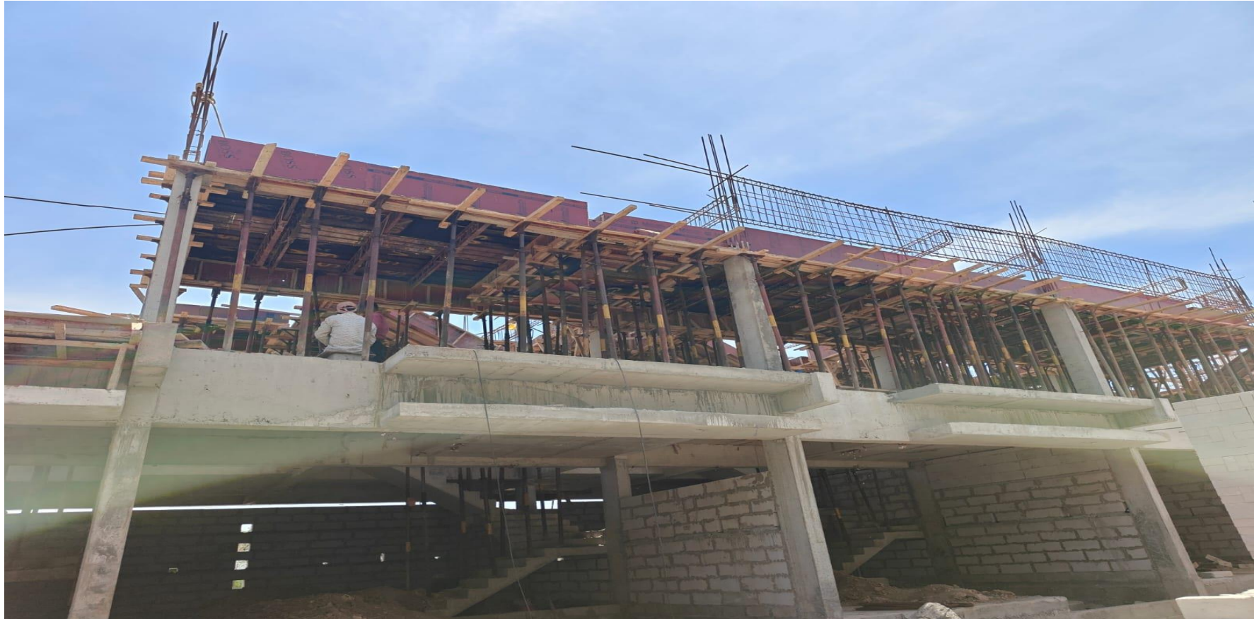
Villa No 94 To 96–FF Roof Slab Beam Reinforcement Work In Progress
