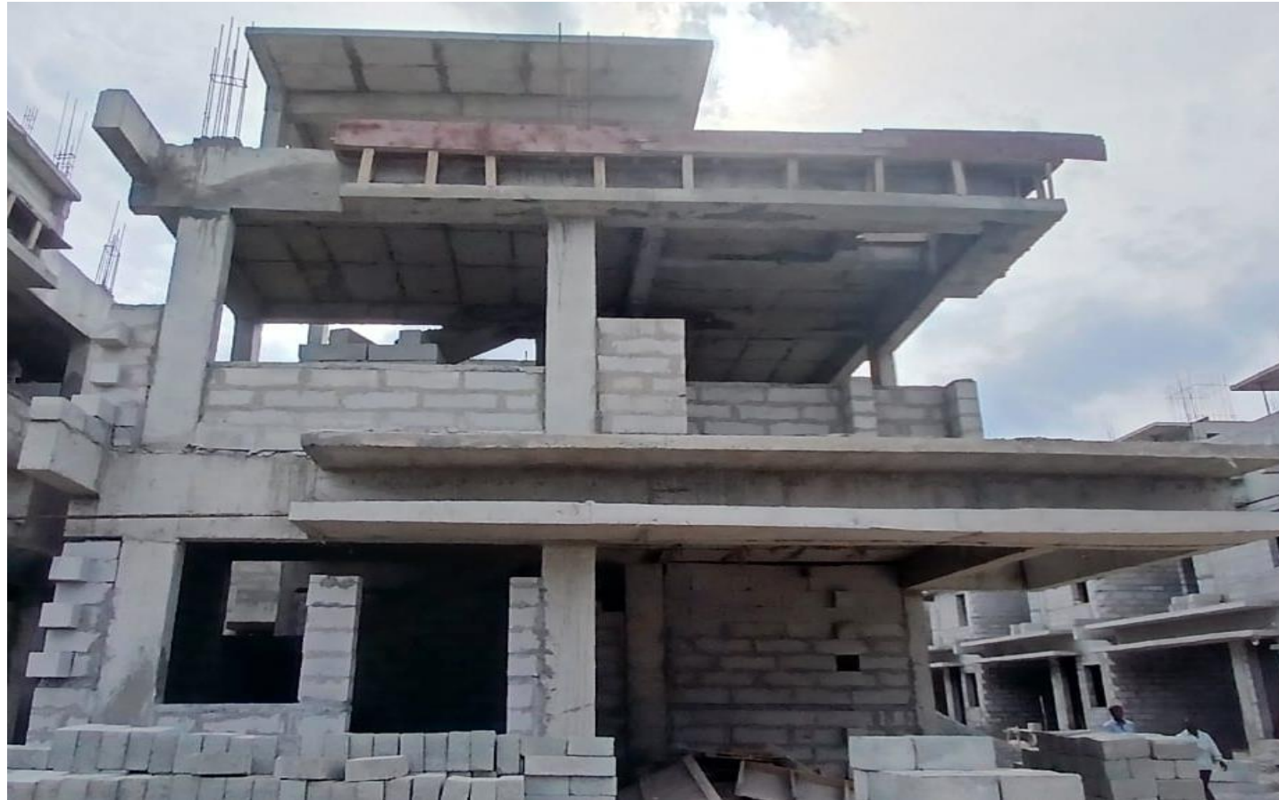
Villa No-55 GF&FF Block Work In Progress
