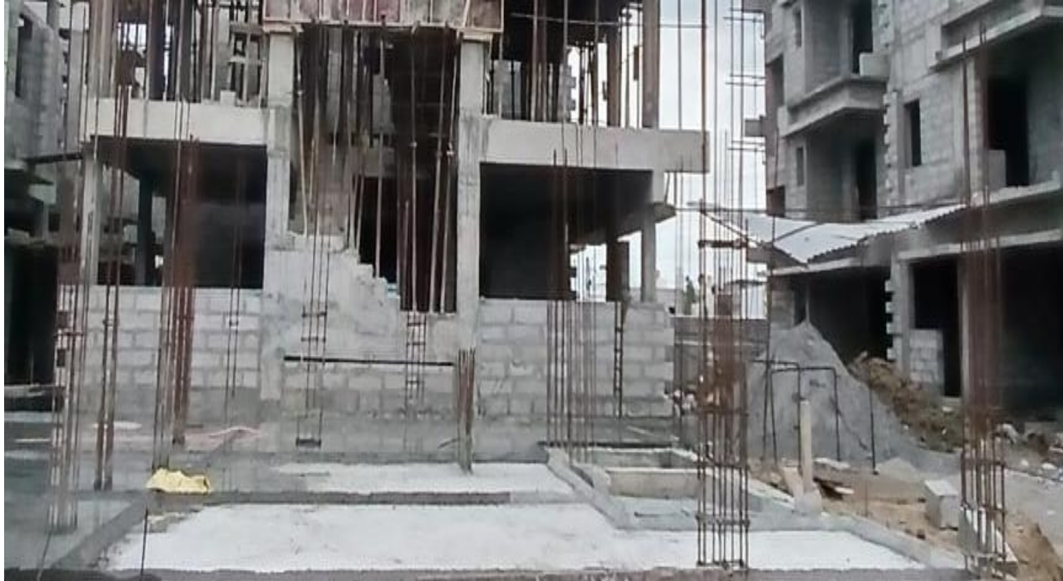
Villa No 34 – GF Floor PCC Work Completed
