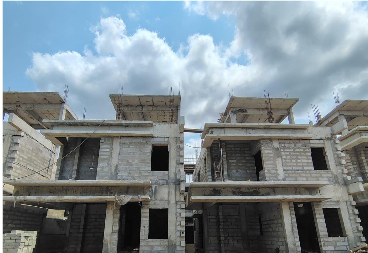
Villa No 49&50- Parapet Wall Column Reinforcement Work In Progress
