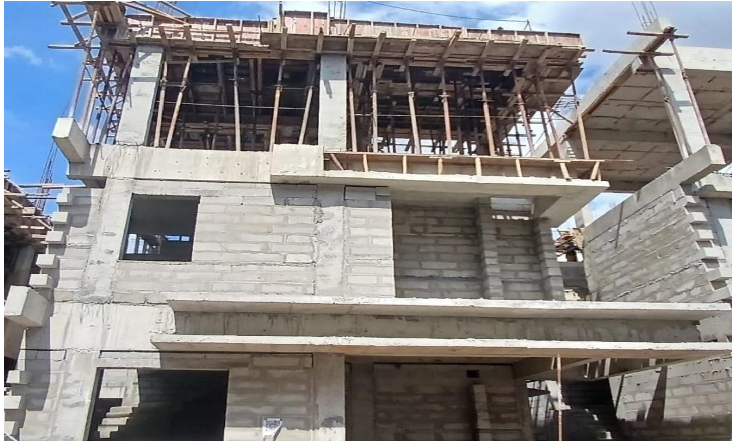
Villa No 37 –SF Roof Slab Concrete Pouring Work Completed
