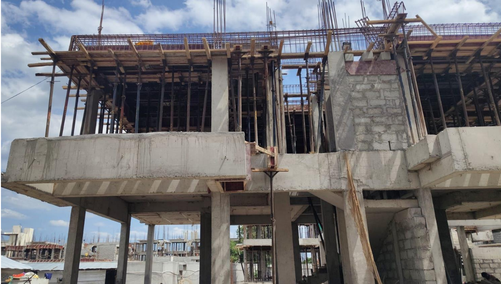
Villa No 104–FF Roof Slab Reinforcement Work Progress
