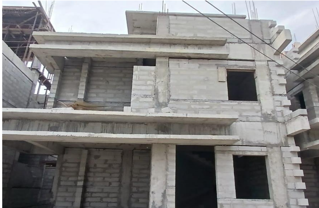
Villa No-65 Parapet Wall Block Work In Progress
