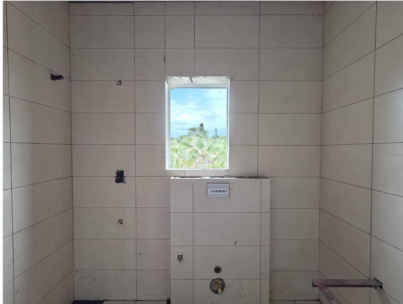
Villa No 9 – FF bedroom toilet wall tile laying work in progress
