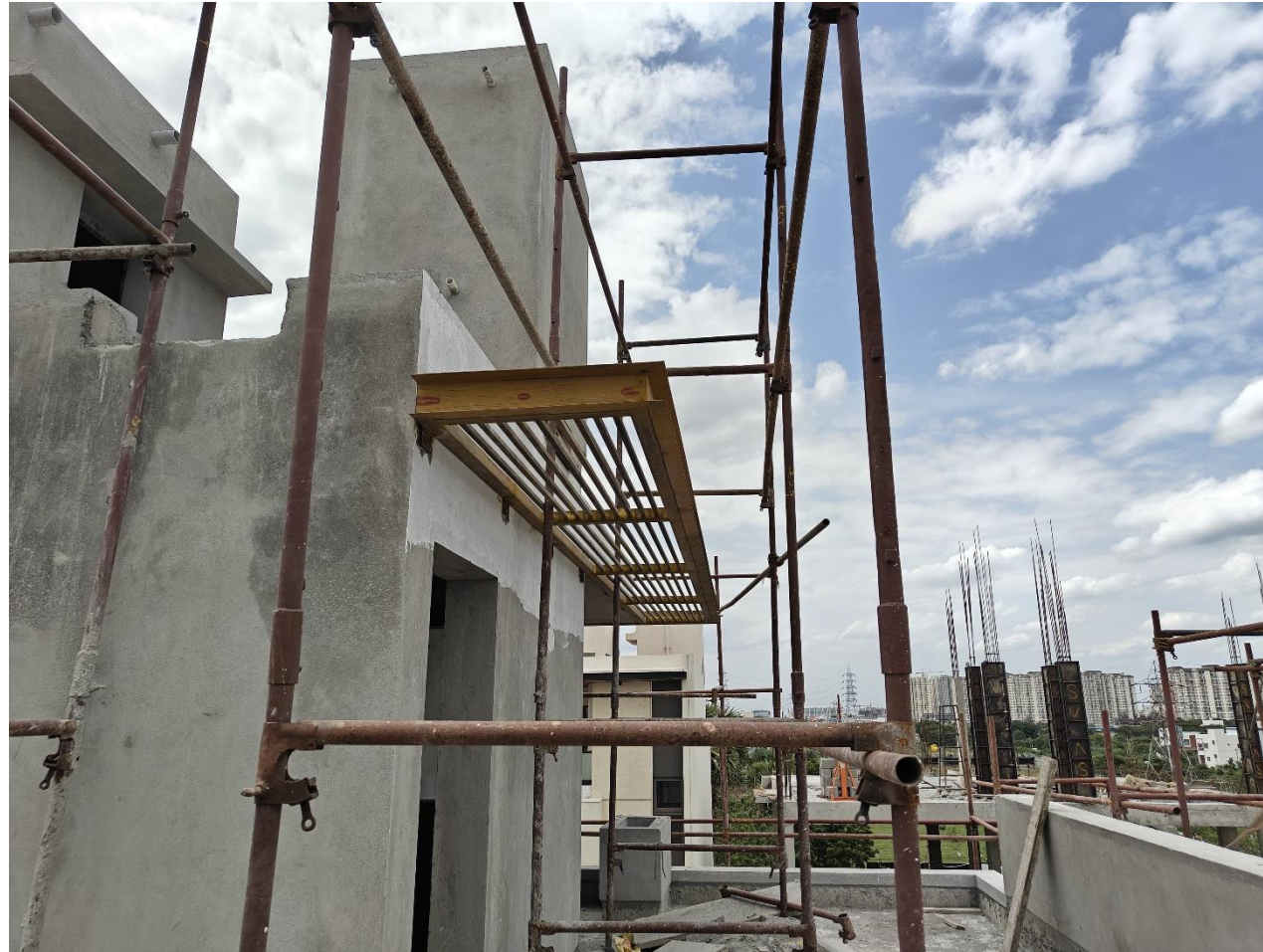
Villa No 6 – Terrace area M.S Percola fixing work in progress
