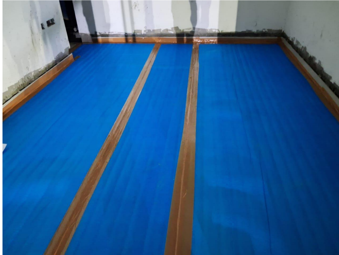
Villa No 5 – FF bedroom tile protection work after tile laying
