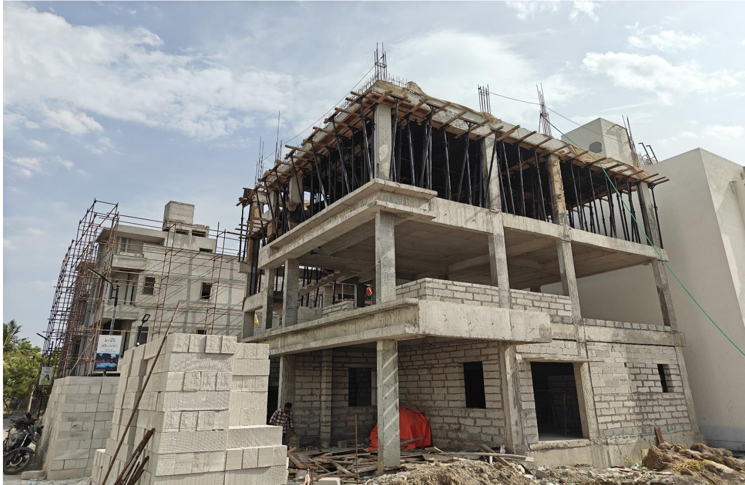
Villa No 17 – SF Roof slab reinforcement work in progress
