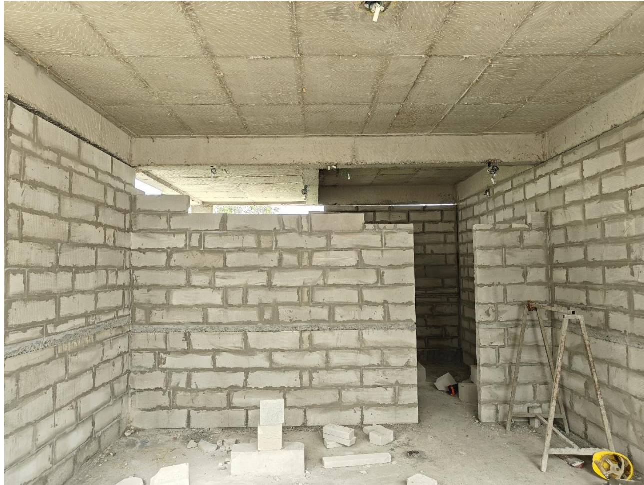
Villa No 17 – FF Bedroom blockwork in progress
