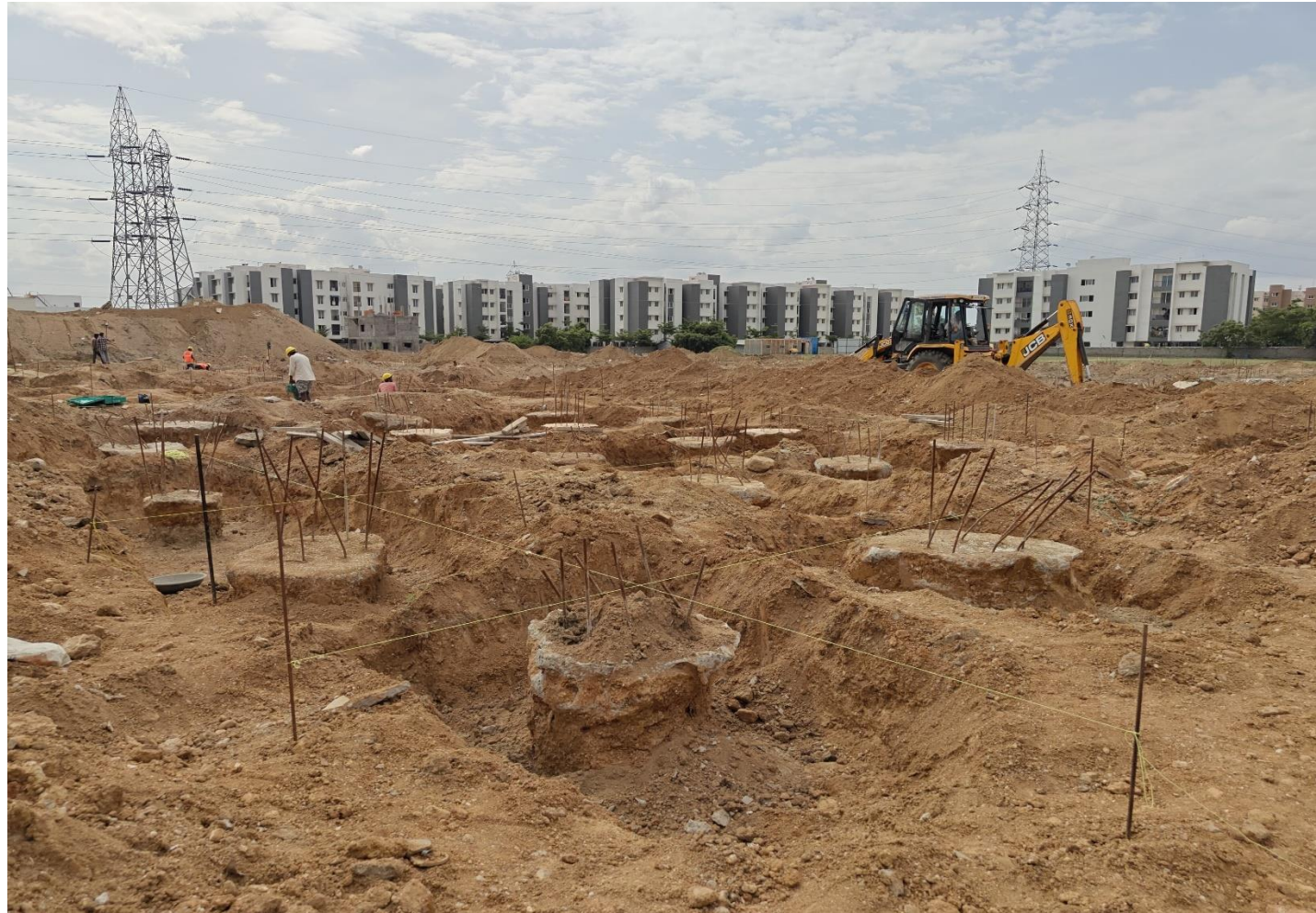
Phase 2 – villa no 53 Earth work for pile cap pcc preparation work in progress
