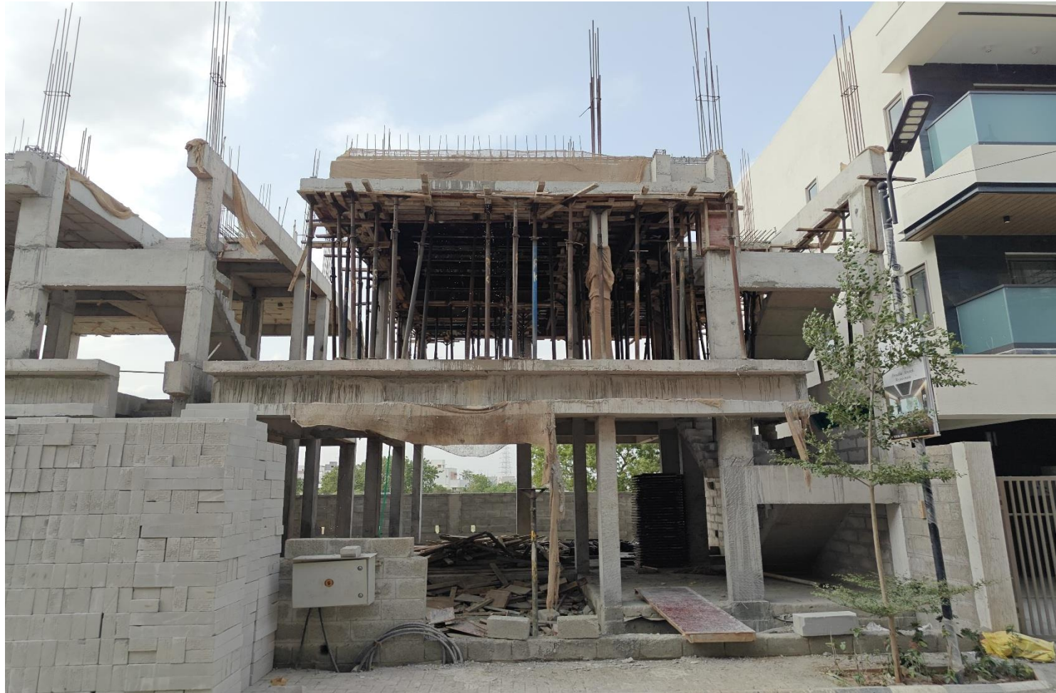
Villa No 15 – FF Roof slab concreting work completed
