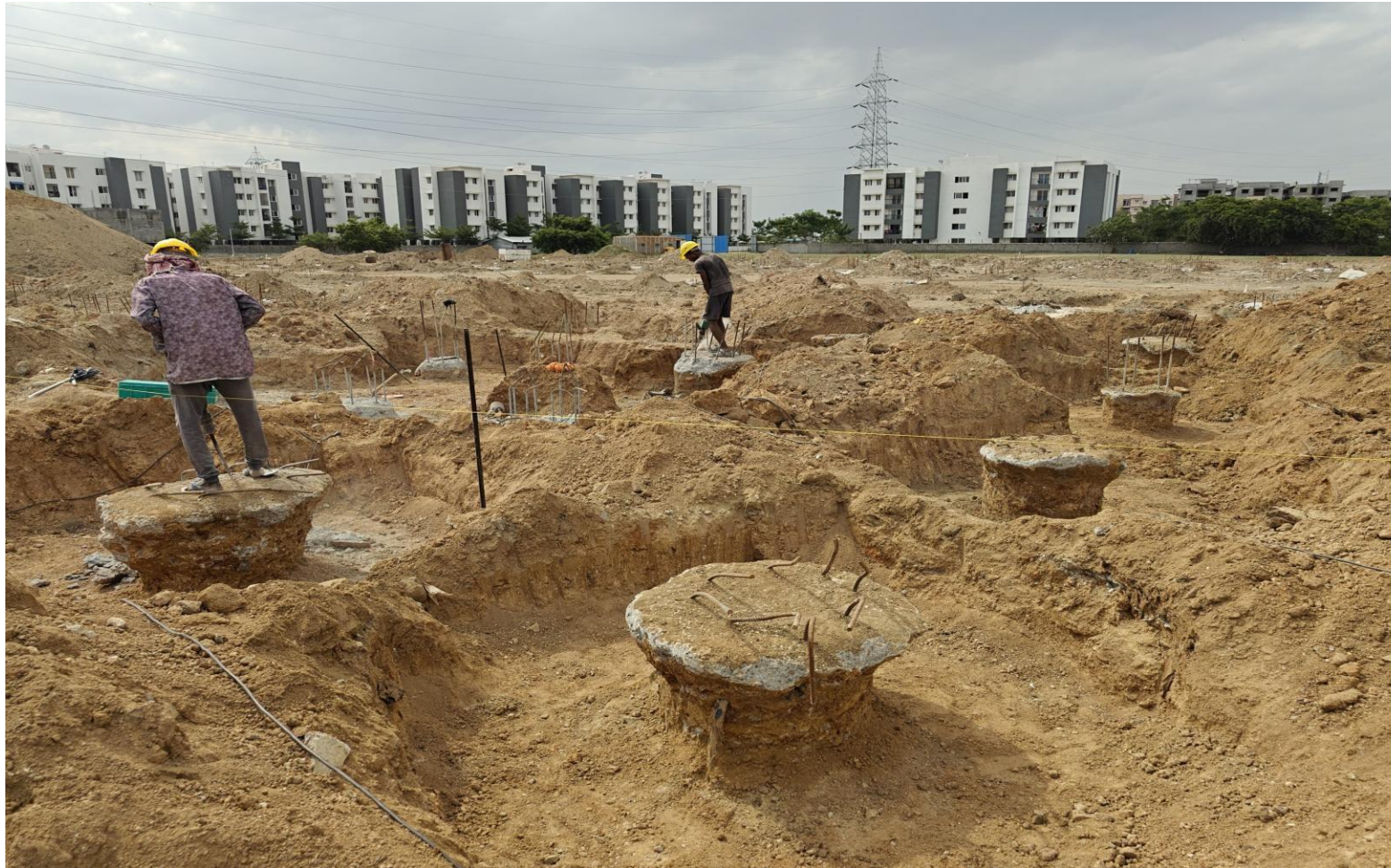
Phase 2 – villa no 51 - pile cap preparation work in progress
