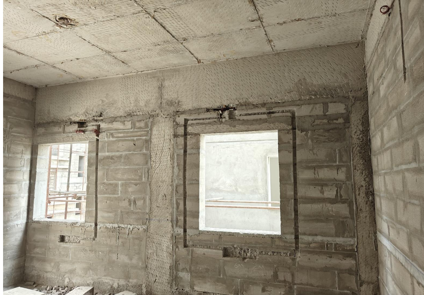
Villa No 13– FF Bedroom electrical wall chasing work in progress
