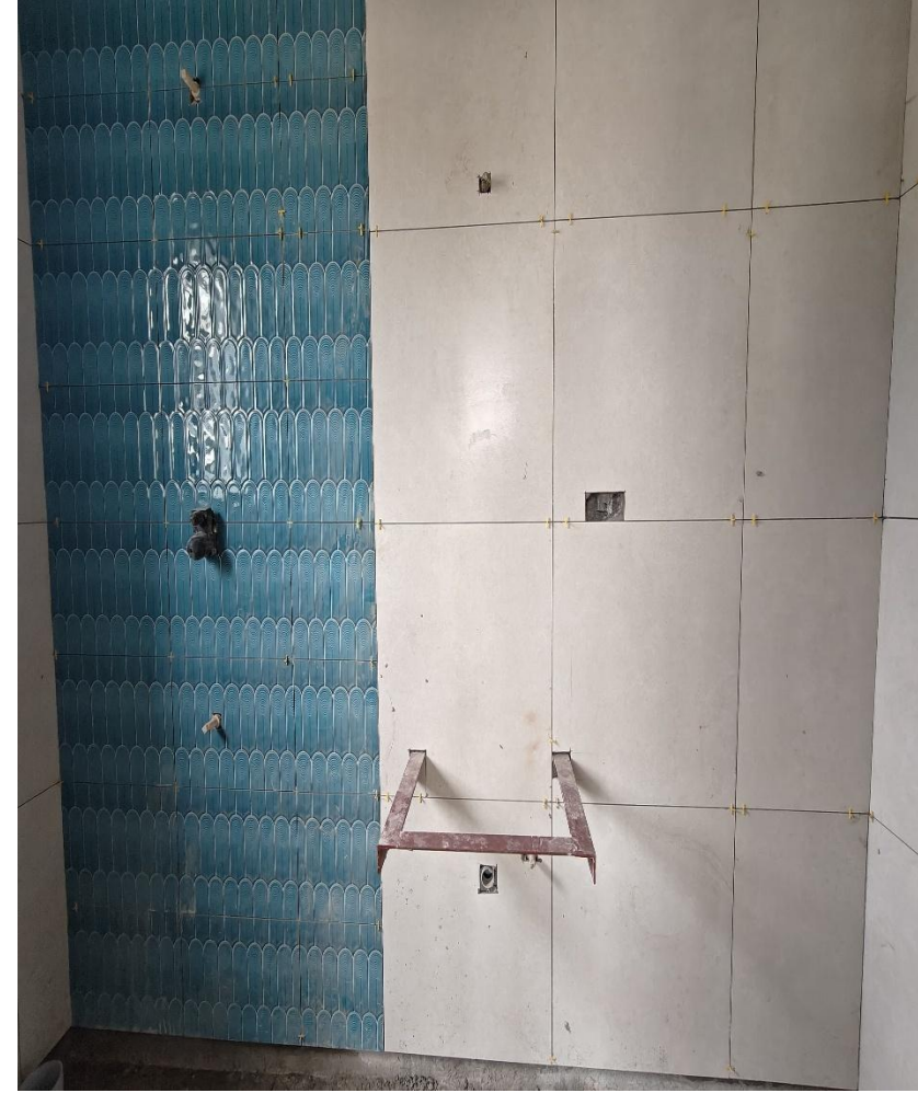
Villa No 5 – SF bedroom toilet wall tile laying work in progress
