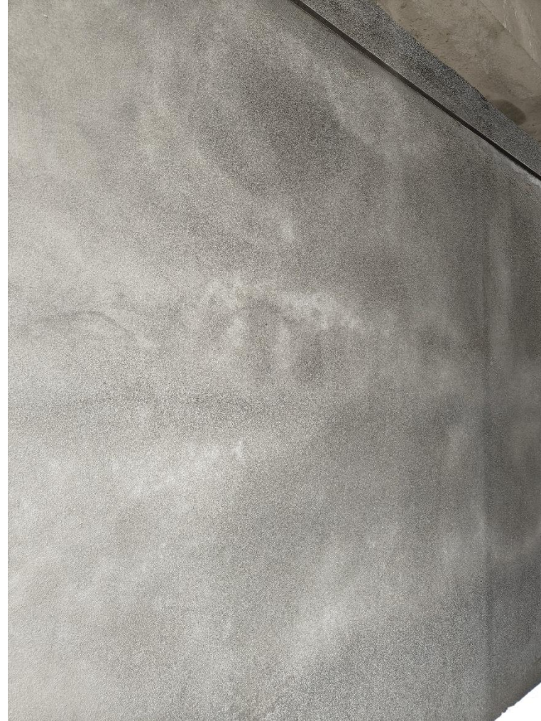
Villa No 7- Westside external wall 2 nd coat plastering work in progress
