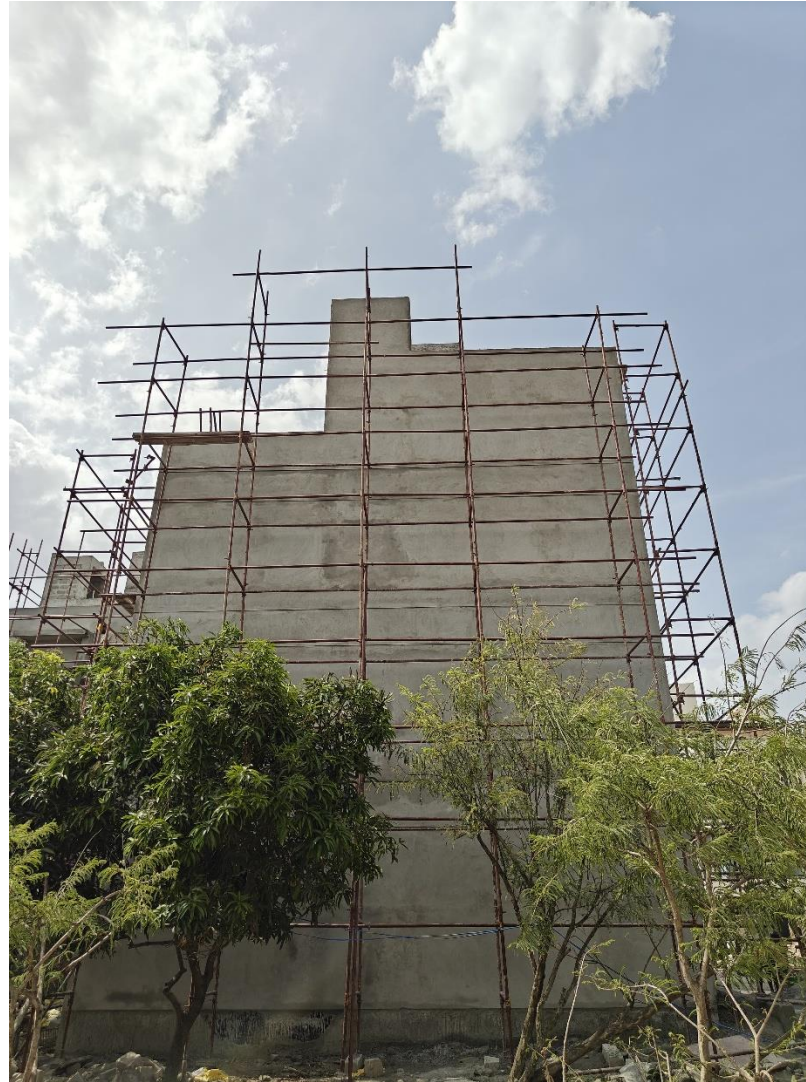
Villa No 4 South side external plastering in work
