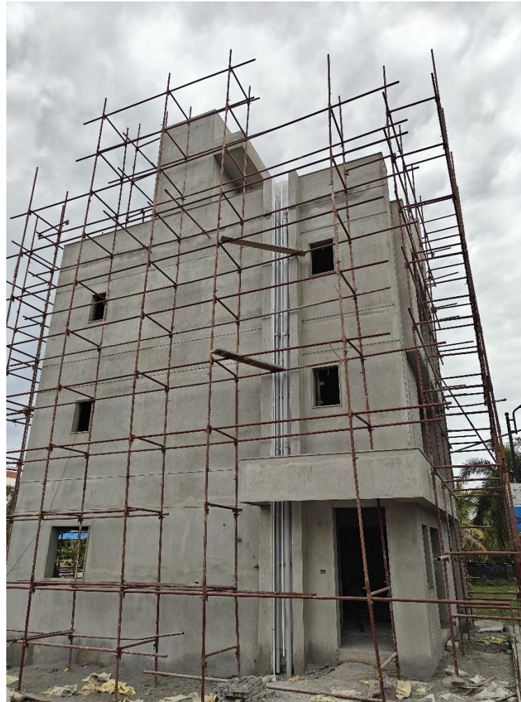
Villa No 3- Northside plumbing shaft pipeline laying work in progress
