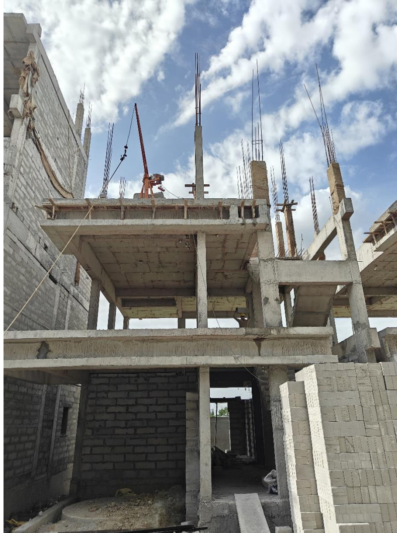
Villa No 14– SF column concreting work completed
