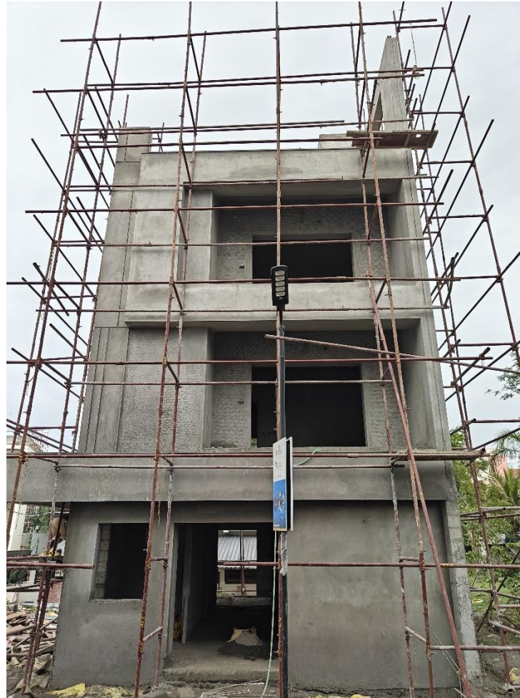
Villa No 3 – Front Elevation plastering work in progress
