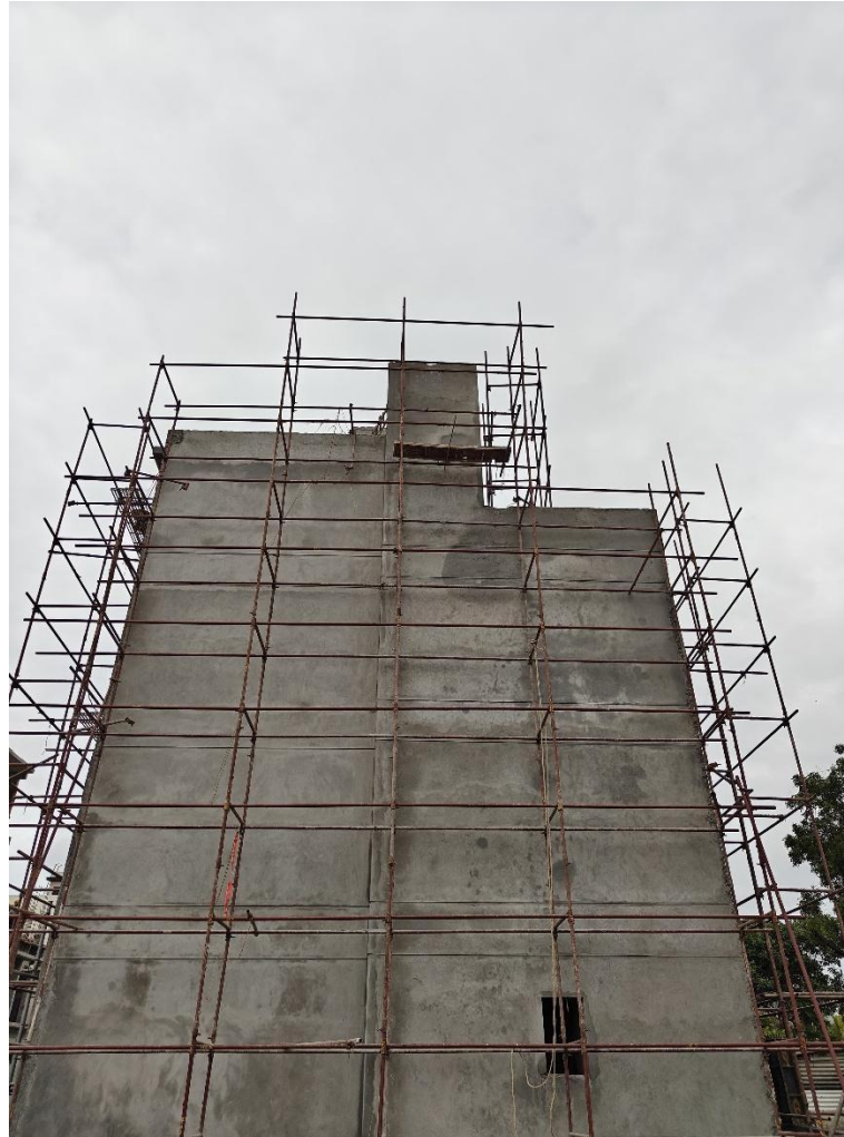
Villa No 11- Westside external plastering work in progress
