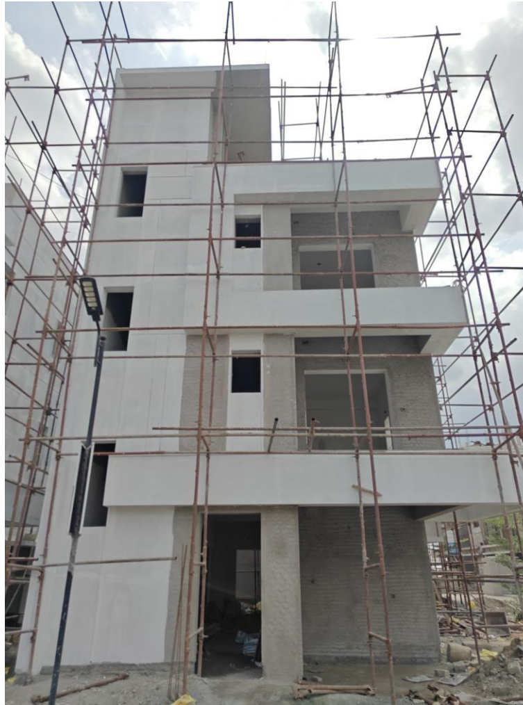
Villa No 5 - External wall primer coat applying work in progress
