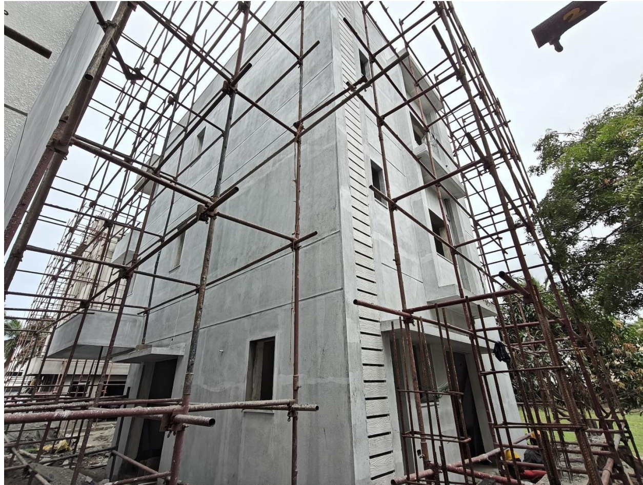
Villa No 4 – Backside plumbing Shaft Shera plank fixing work in progress
