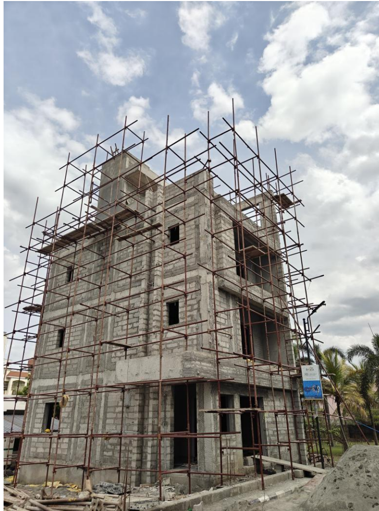
Villa No 3 - Northwest corner view
