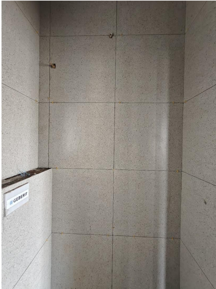
Villa No 5 – FF bedroom toilet wall tile laying work in progress
