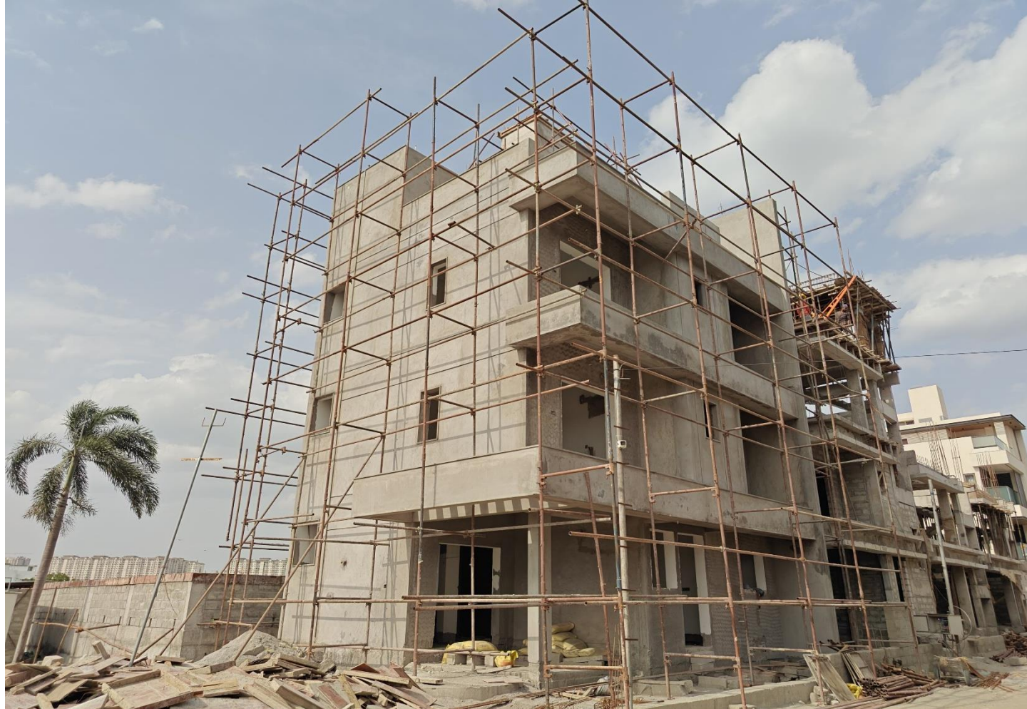
Villa No 12 – External plastering work in progress
