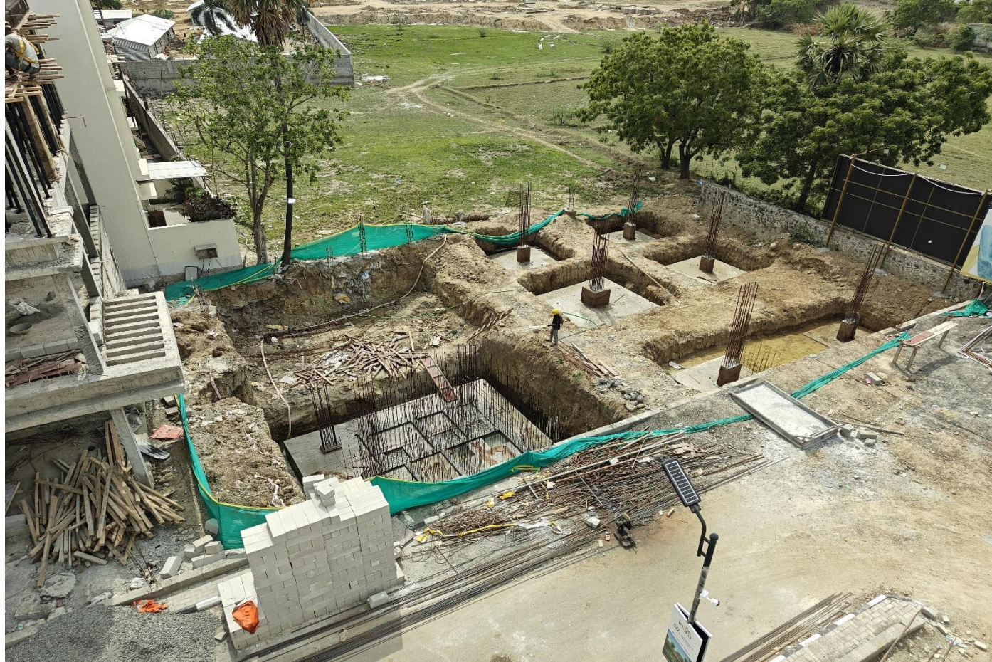
Clubhouse sub-structure column concreting work completed
