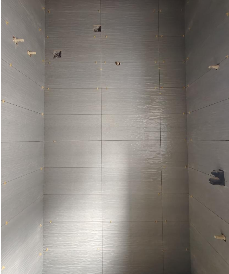
Villa No 5 – SFbedroomtoilet wall tilelaying work in progress
