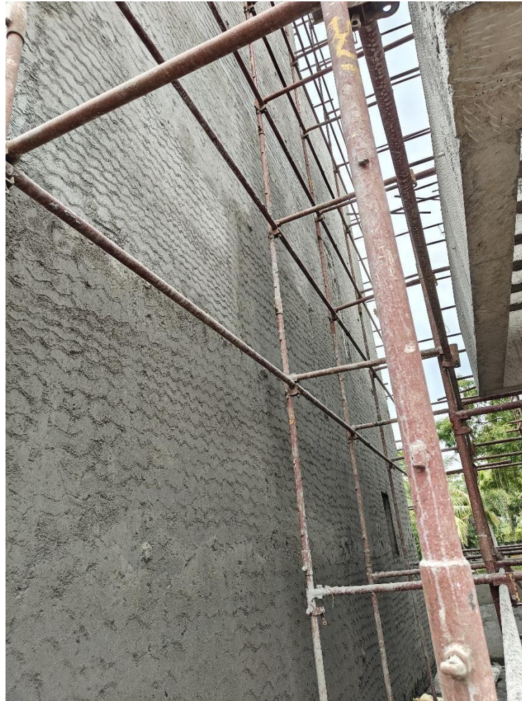
VillaNo 10- Westside external wall 1 st coat rough plastering work in progress
