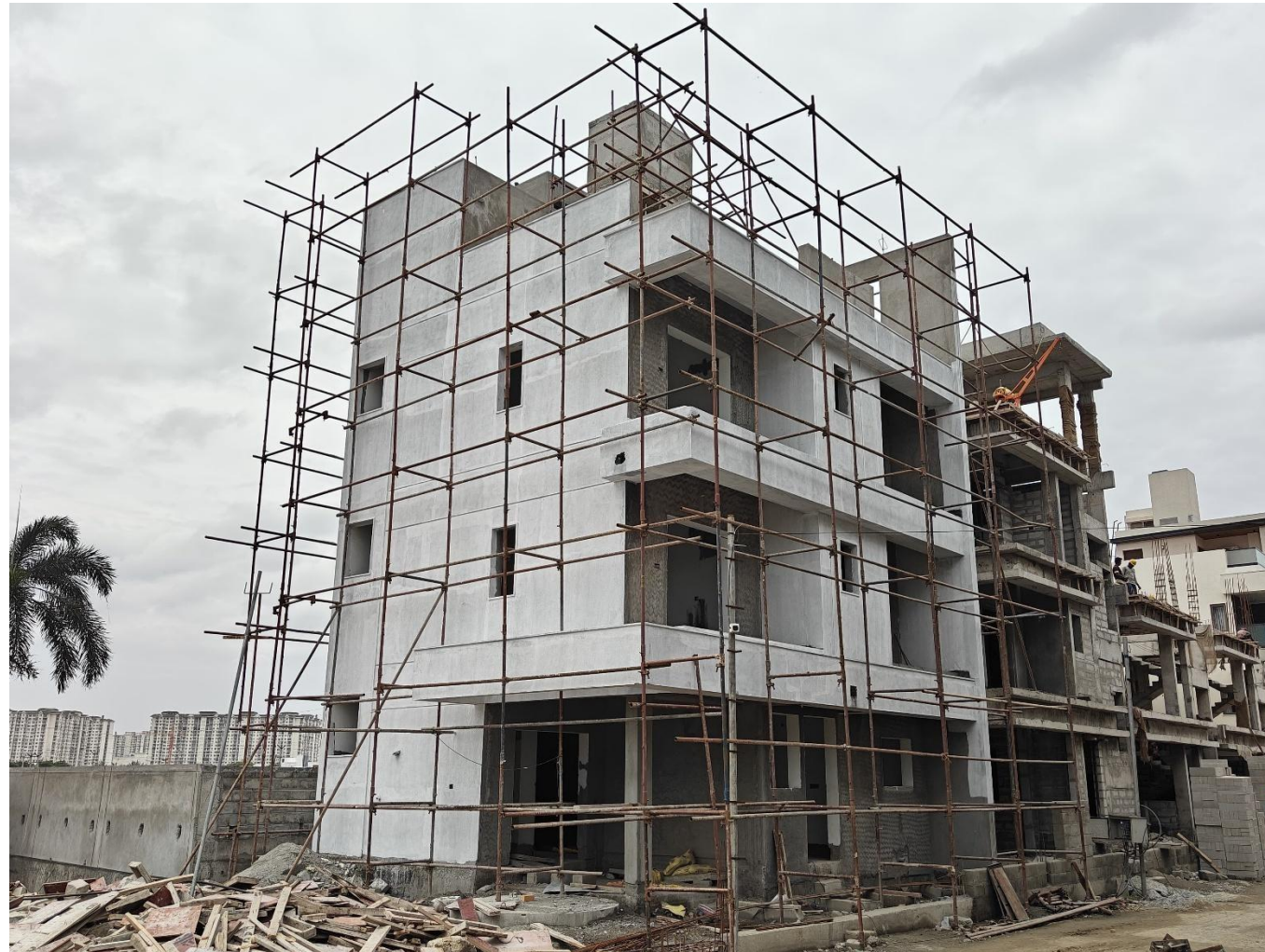
Villa No 12 – External wall primer coat applying work in progress
