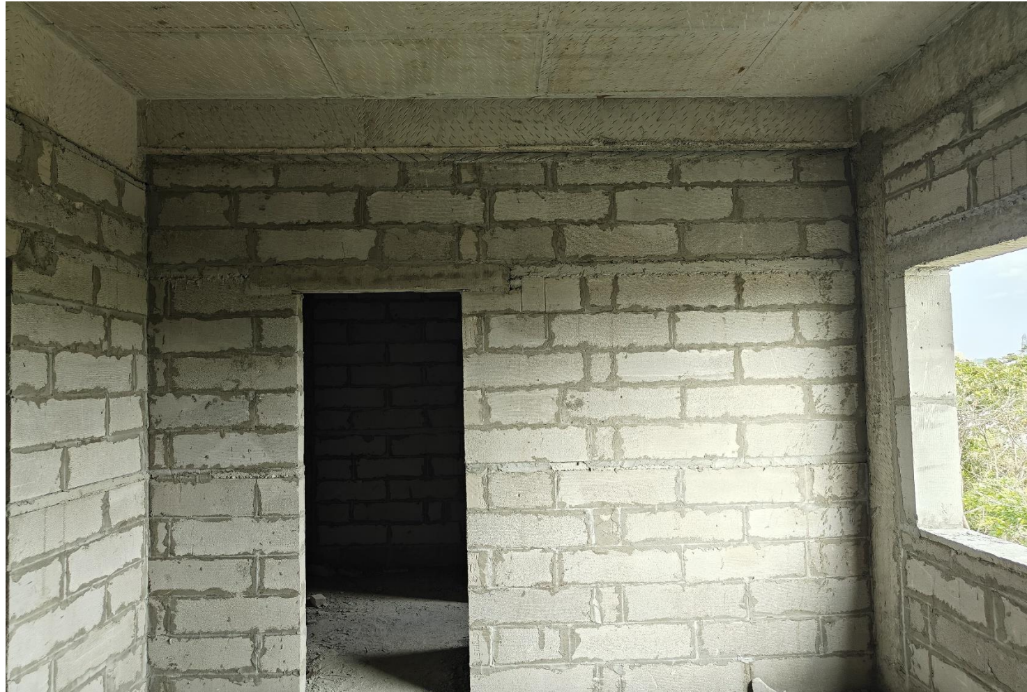
Villa No 8 – SF Bedroom blockwork in progress
