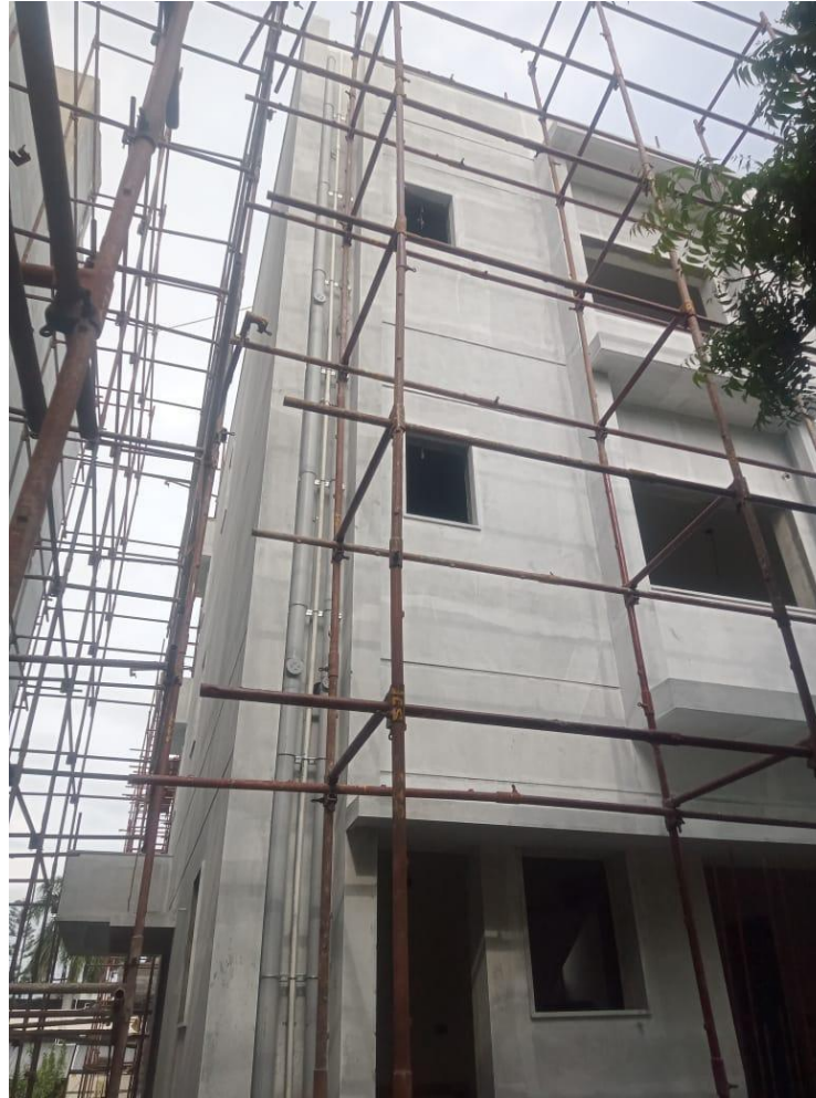
Villa No 5 – Backside plumbing shaft pipeline laying work in progress
