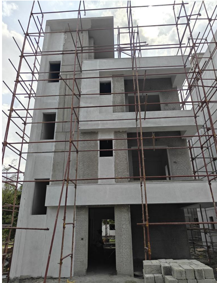
Villa No 4 - External wall primer coat applying work in progress
