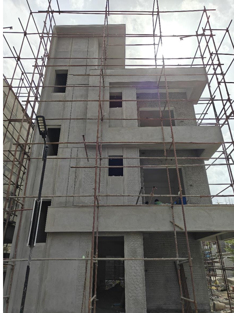
Villa No 5 – Front side Elevation view
