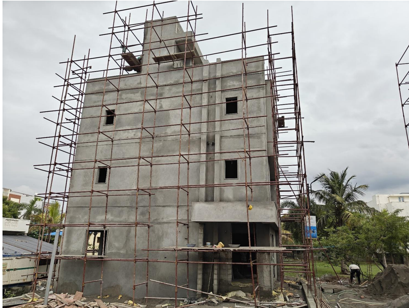
Villa No 3- Northsideexternal wall plastering work in progress
