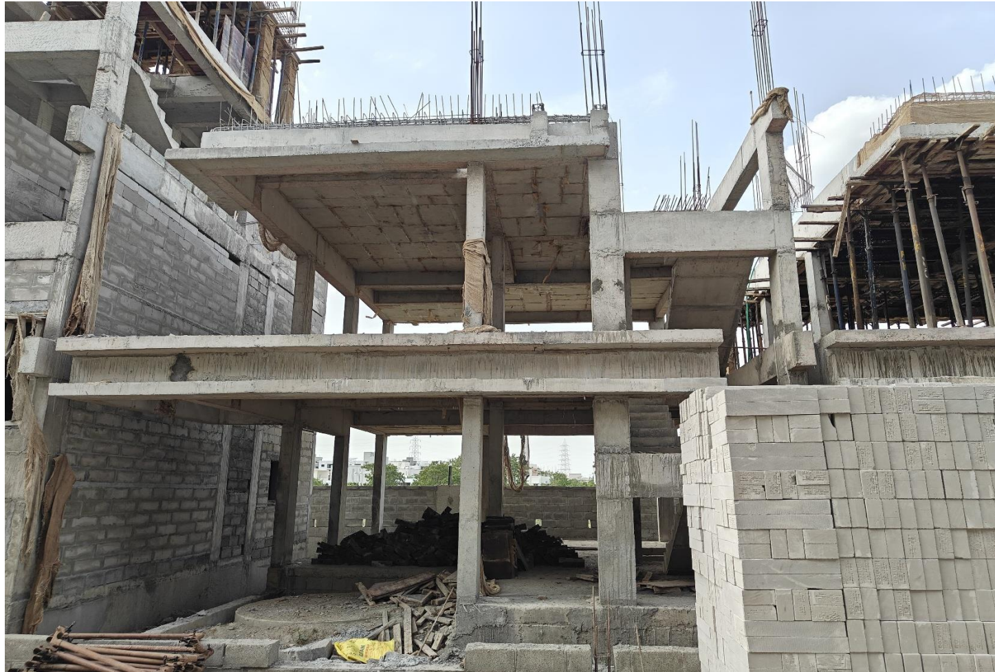
Villa No 14 – FF Roof slab concreting work completed
