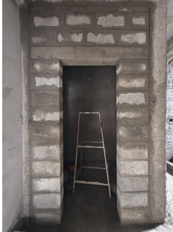
Villa No 7- FF lift elevation blockwork in progress
