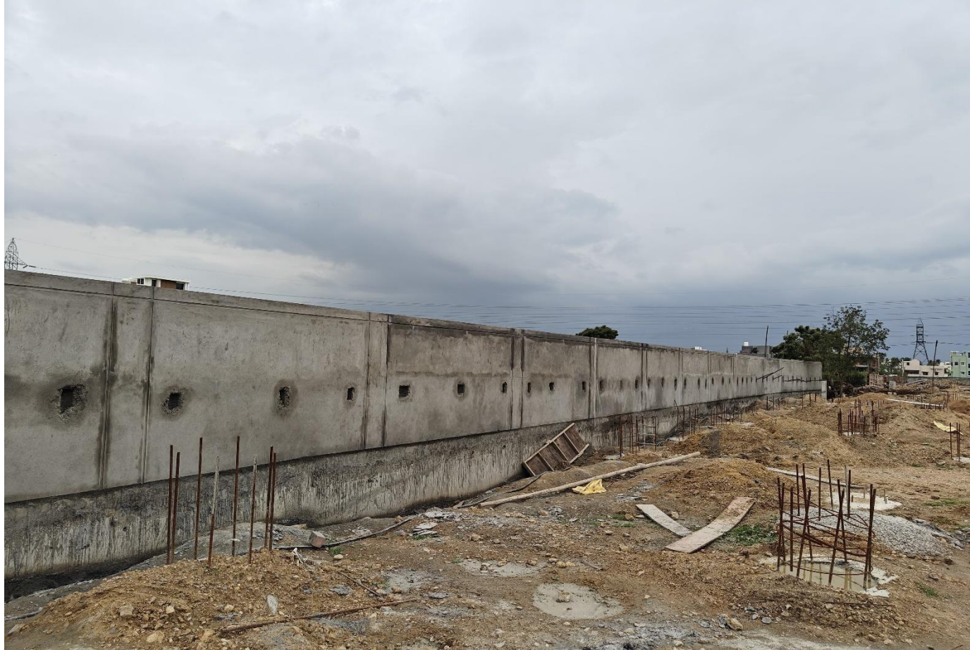
Phase 1 - South Side Compound wall internal plastering work in progress
