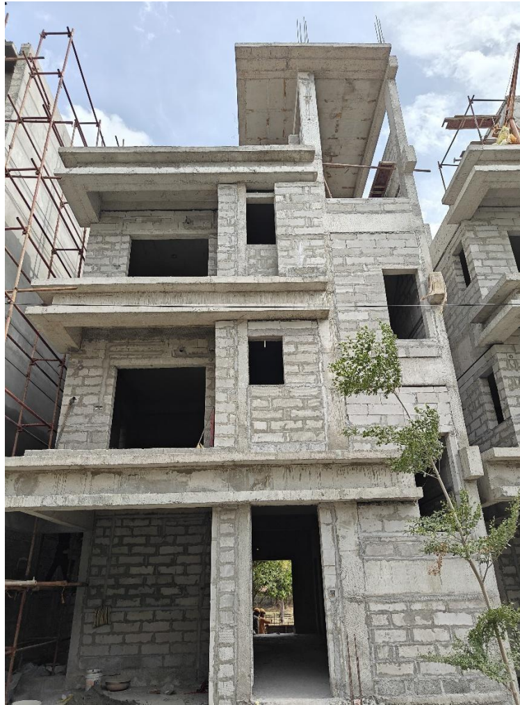
Villa No 7- FrontElevationview
