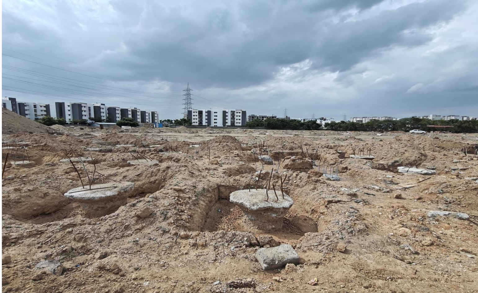
Phase 2 – villa no 48 to 51 pile cap preparation work in progress
