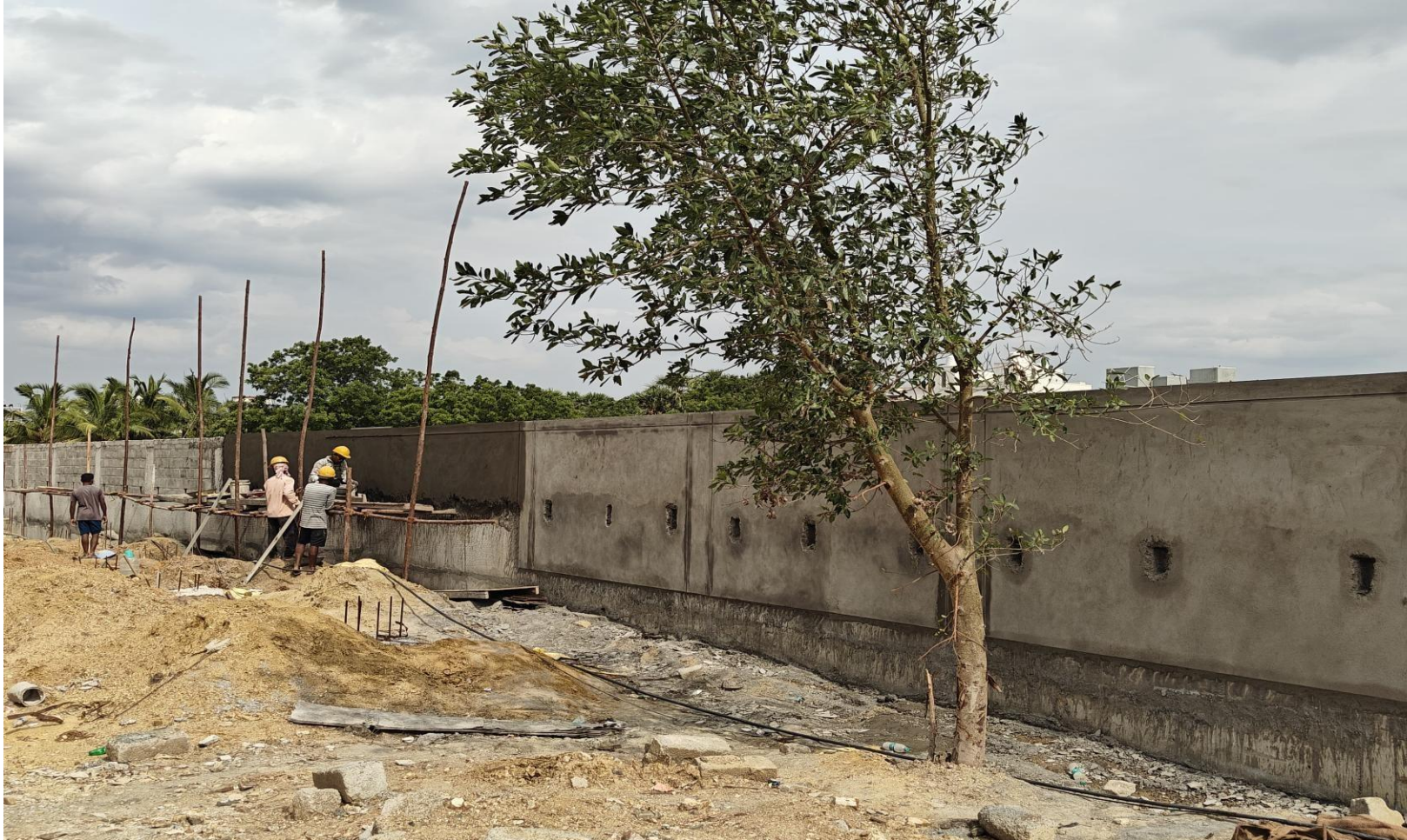
South Side Compound wall internal plastering work in progress
