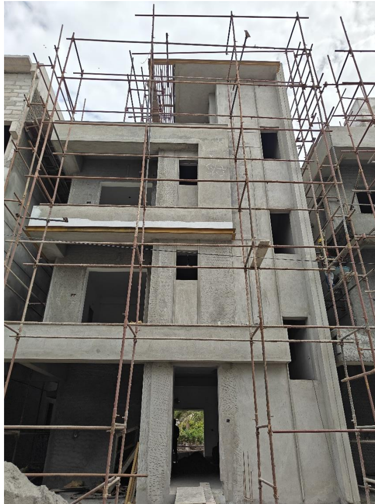
Villa No 9 –Front Elevation view MS ‘C’ Channel fixing work in progress
