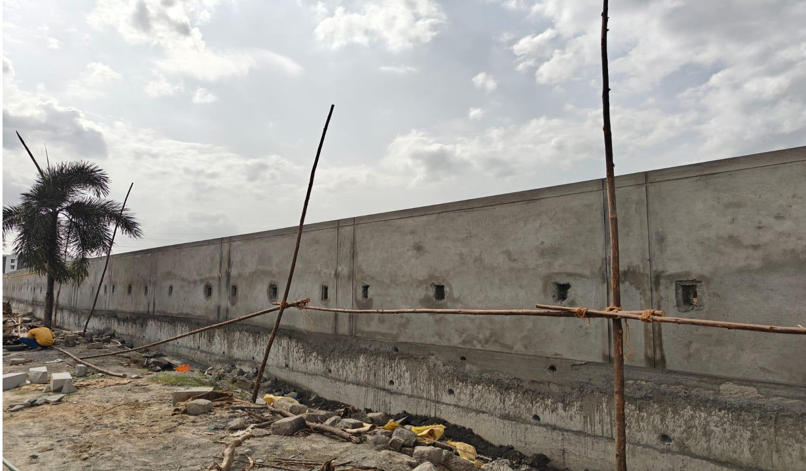
North Side Compound wall internal plastering in progress
