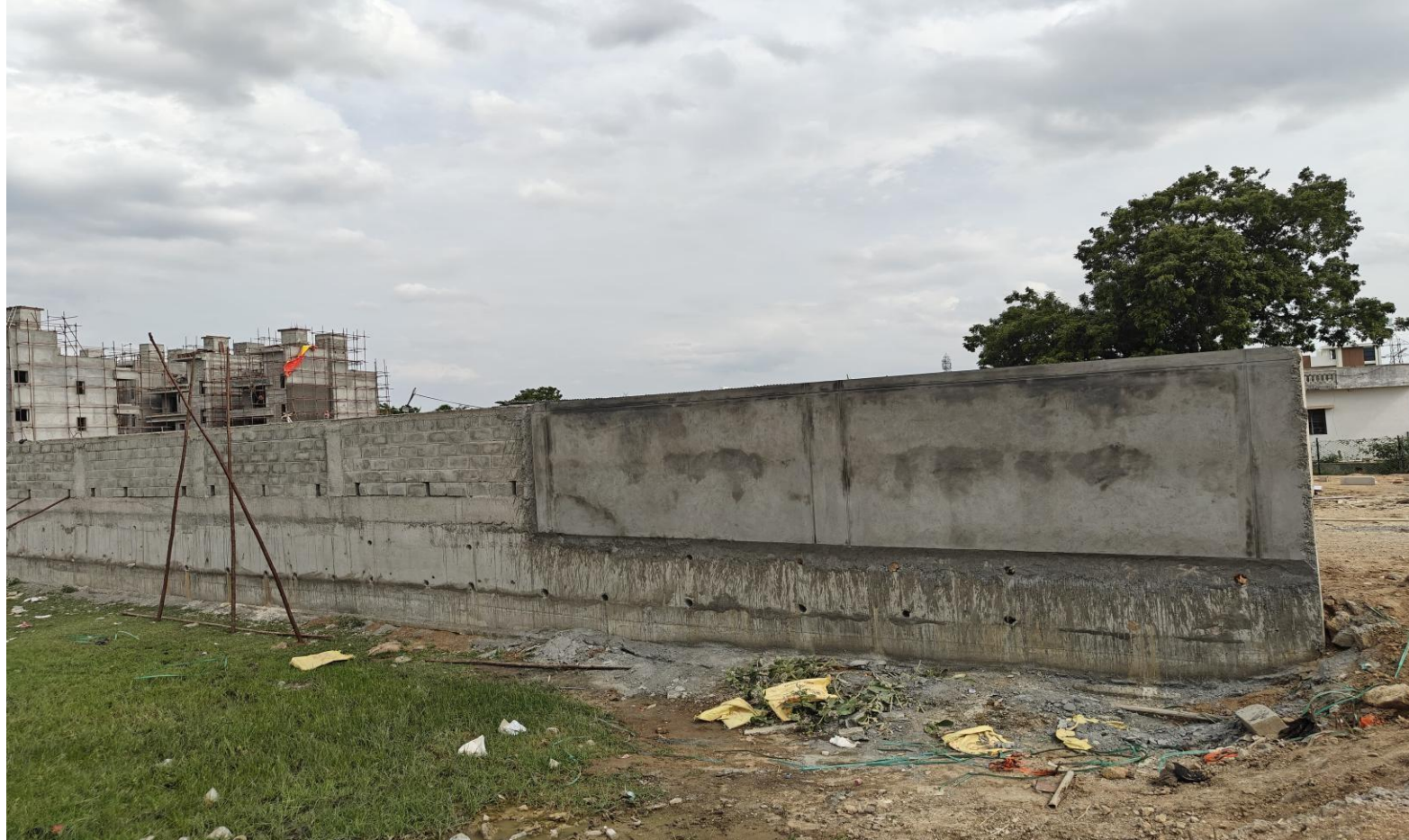
North Side Compound wall External plastering in progress
