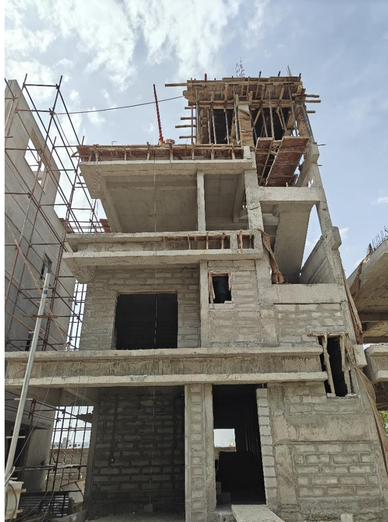
Villa No 13 – Head room Roof slab shuttering work in progress
