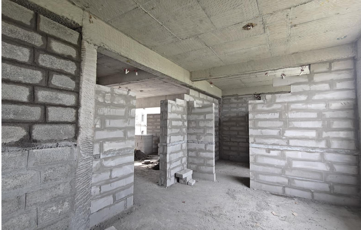
Villa No 13 – SF Bedroom Blockwork in progress
