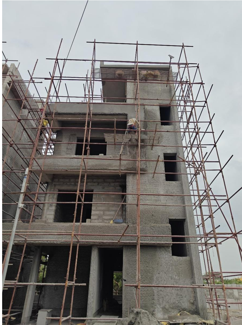
Villa No 11- Front elevation plastering work in progress
