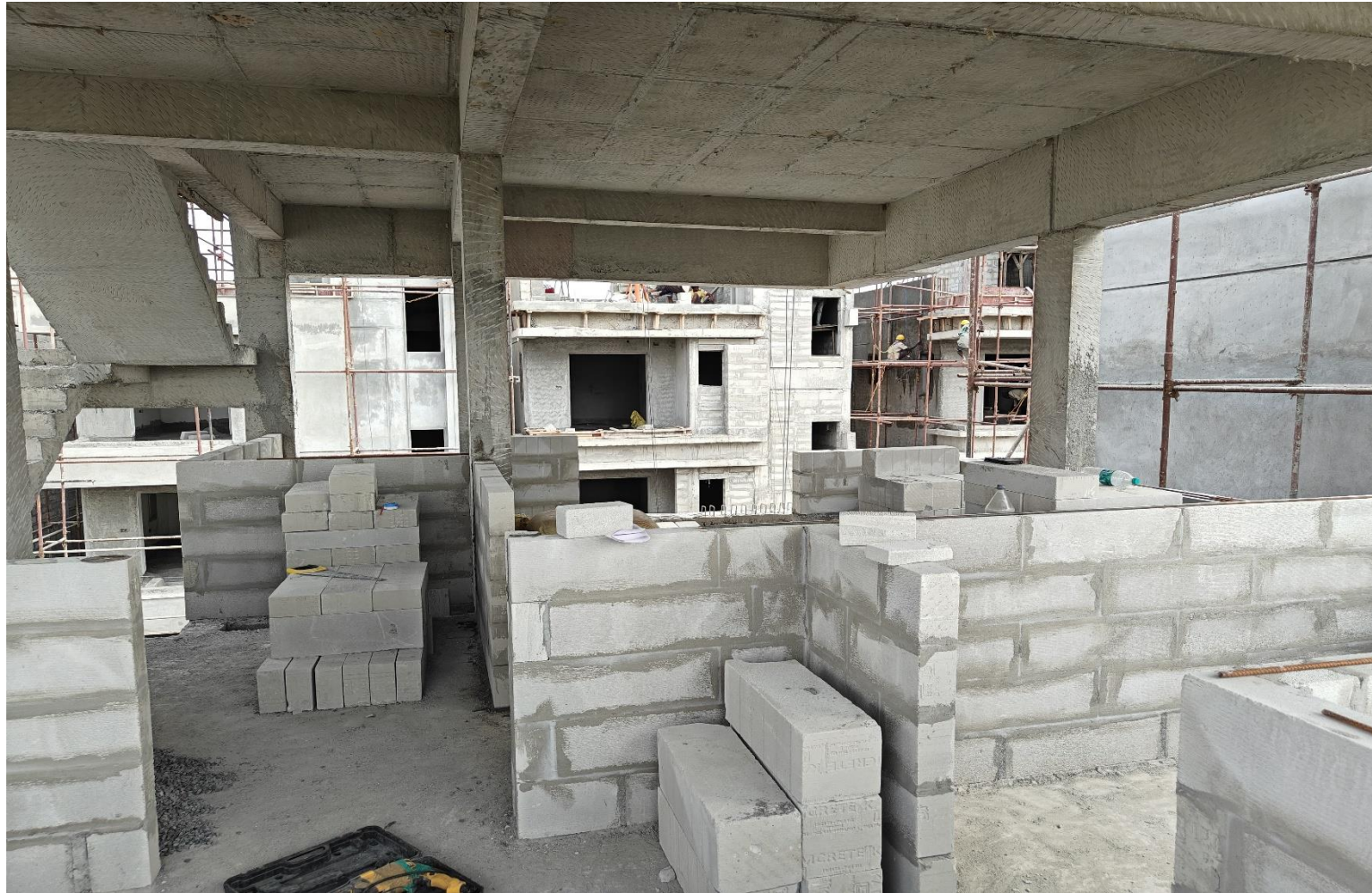
Villa No 13– SF Bedroom Blockwork in progress
