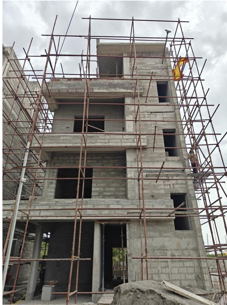
Villa No 11- External scaffolding fixing work in progress
