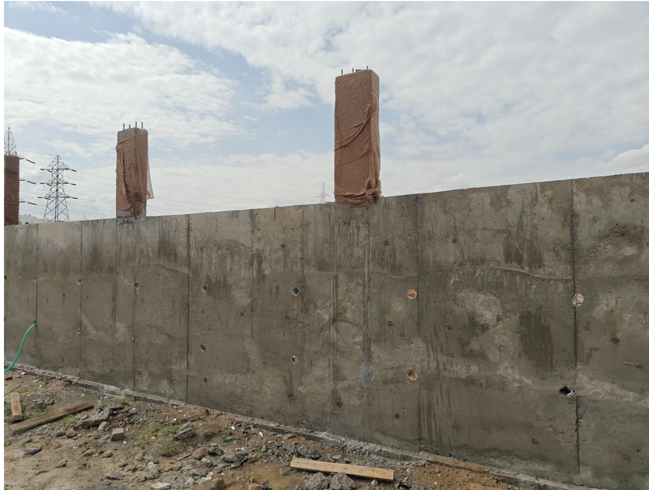
Phase 2 - Southside compound RCC wall concreting work in progress
