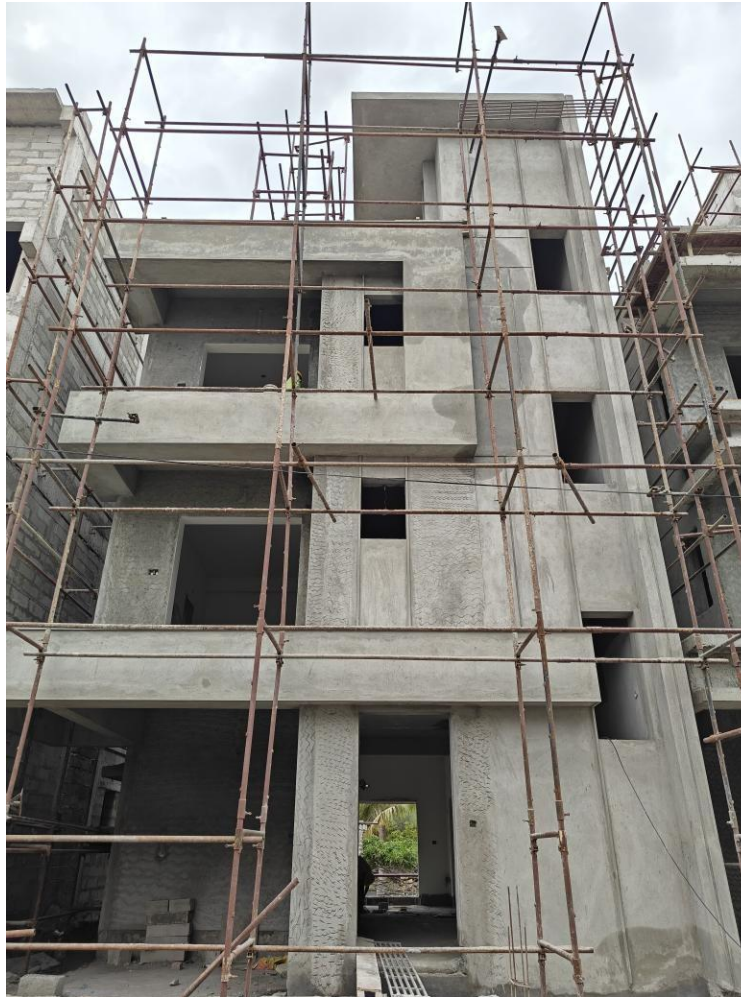
Villa No 9 – Front Elevation external plastering work in progress
