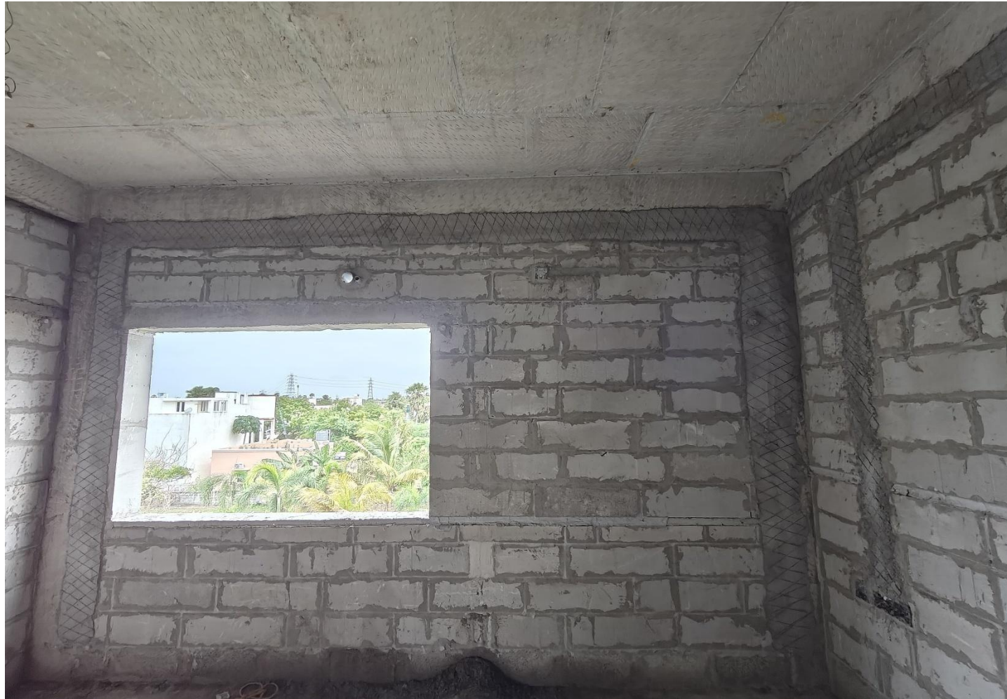
Villa No 8 - FF bedroom internal plastering preparation work in progress
