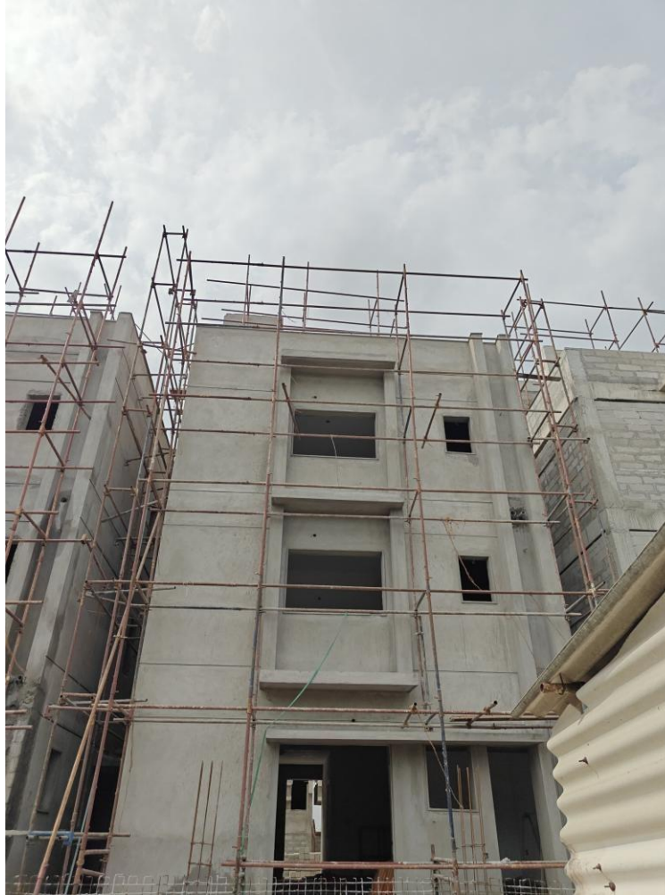
Villa No 9 – Southside external wall plastering work in progress
