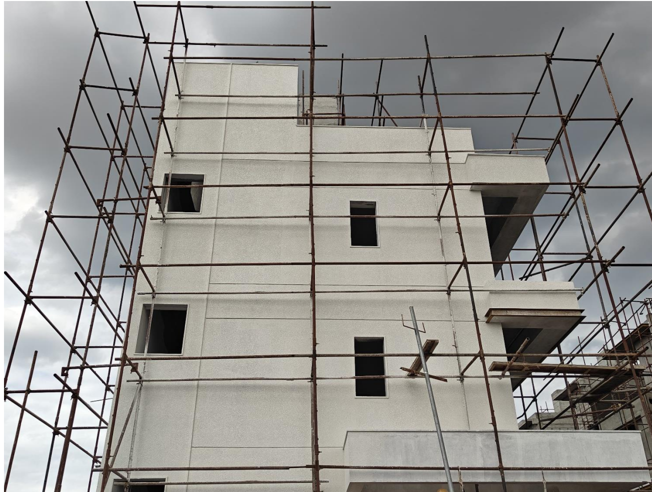
Villa No 12 – External wall pebble texture applying work in progress
