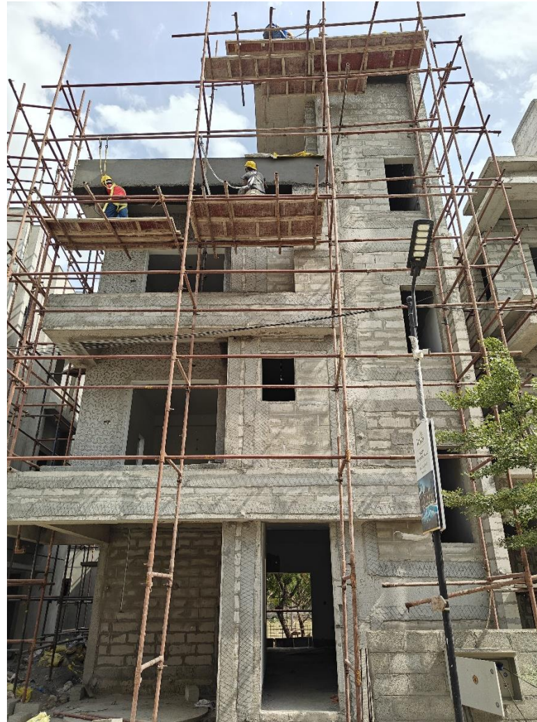
Villa No 6 – Front elevation plastering work in progress
