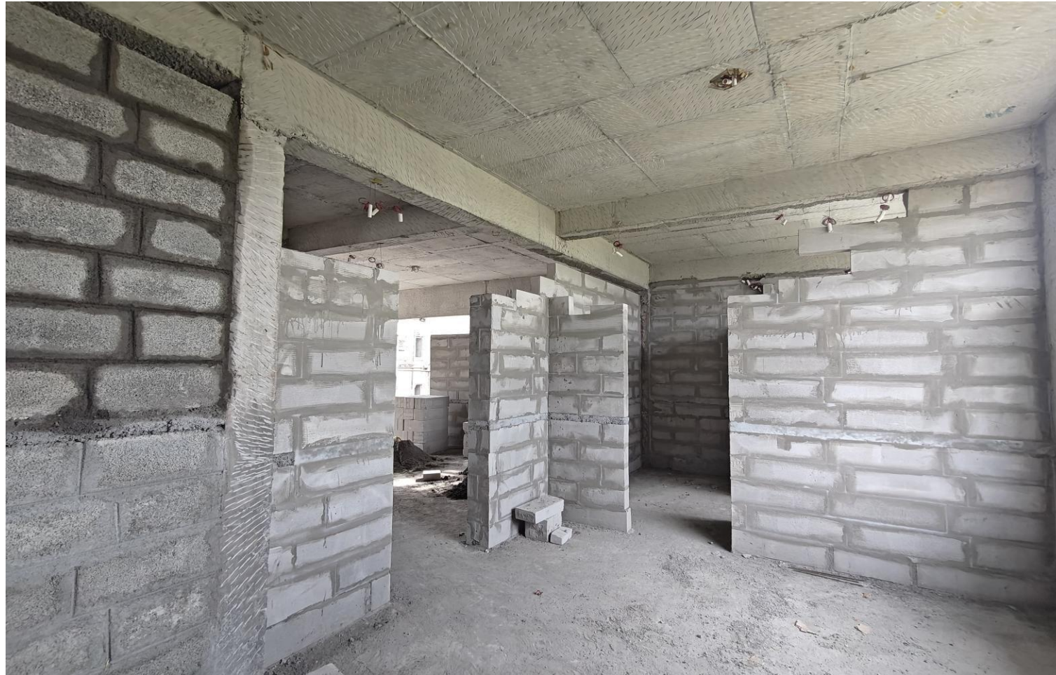
Villa No 13– SF Bedroom block work in progress
