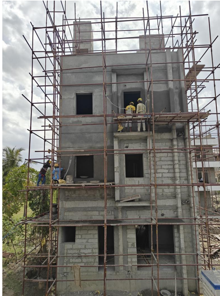
Villa No 3- Eastsideexternal wall plastering work in progress
