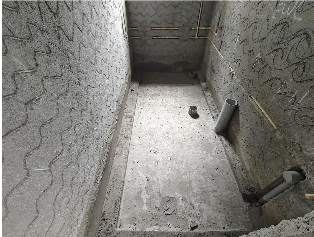
Villa No 3- GF Powder toilet screed concrete pouring work completed
