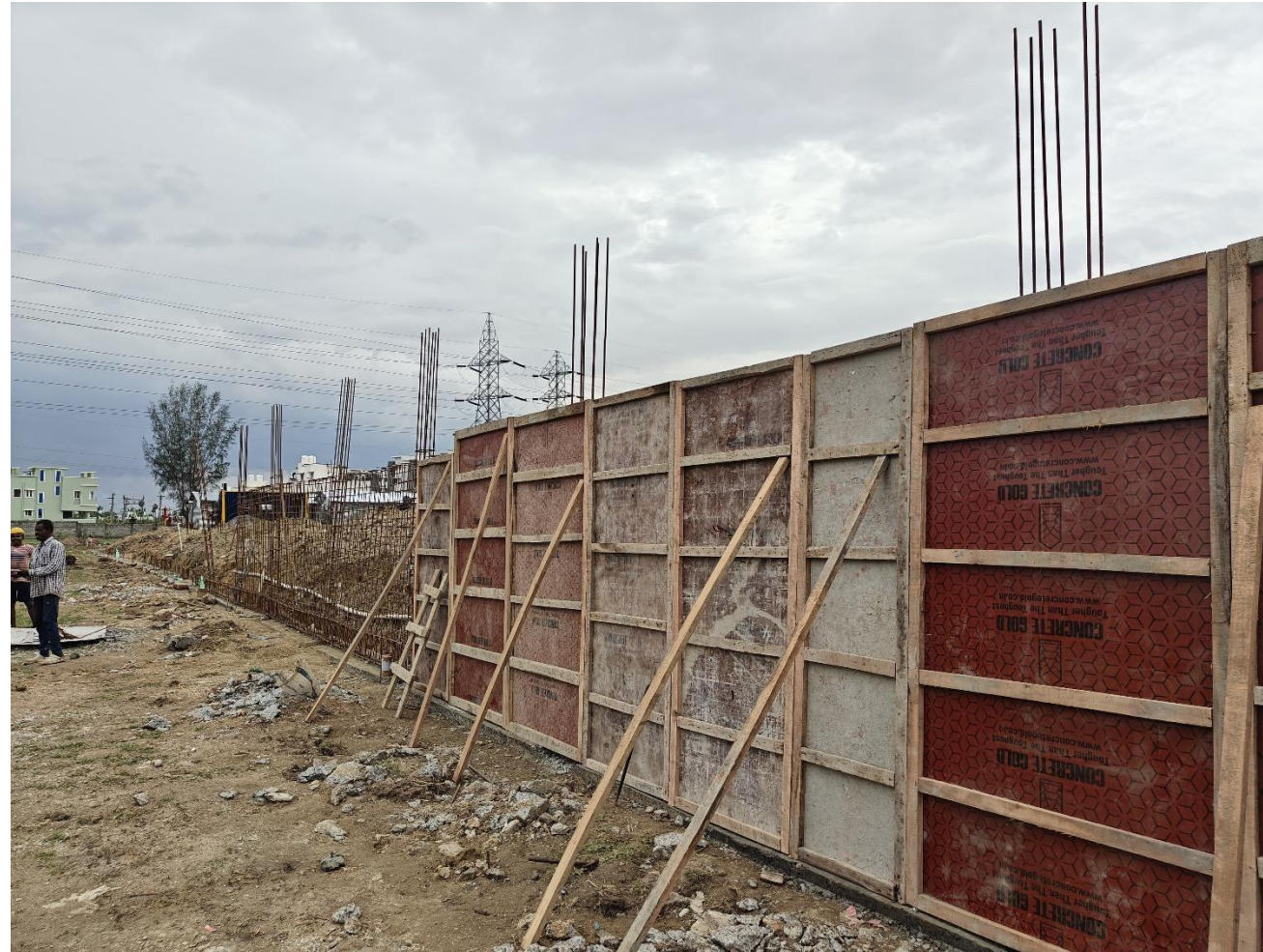
Phase 2 - Southside Ccompound RCC wall shuttering work in progress
