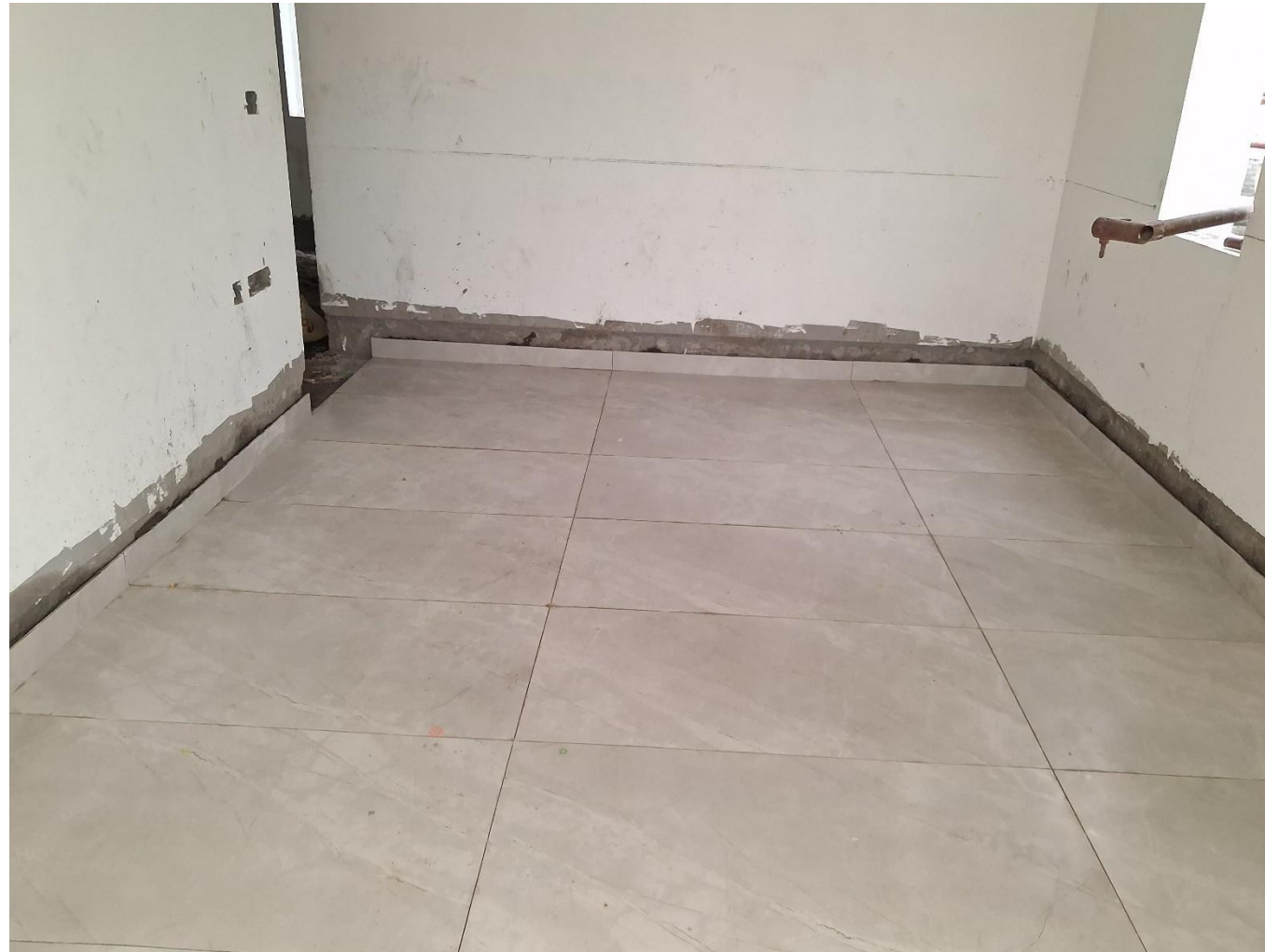
Villa No 5 – SF bedroom flooring tile laying work in progress
