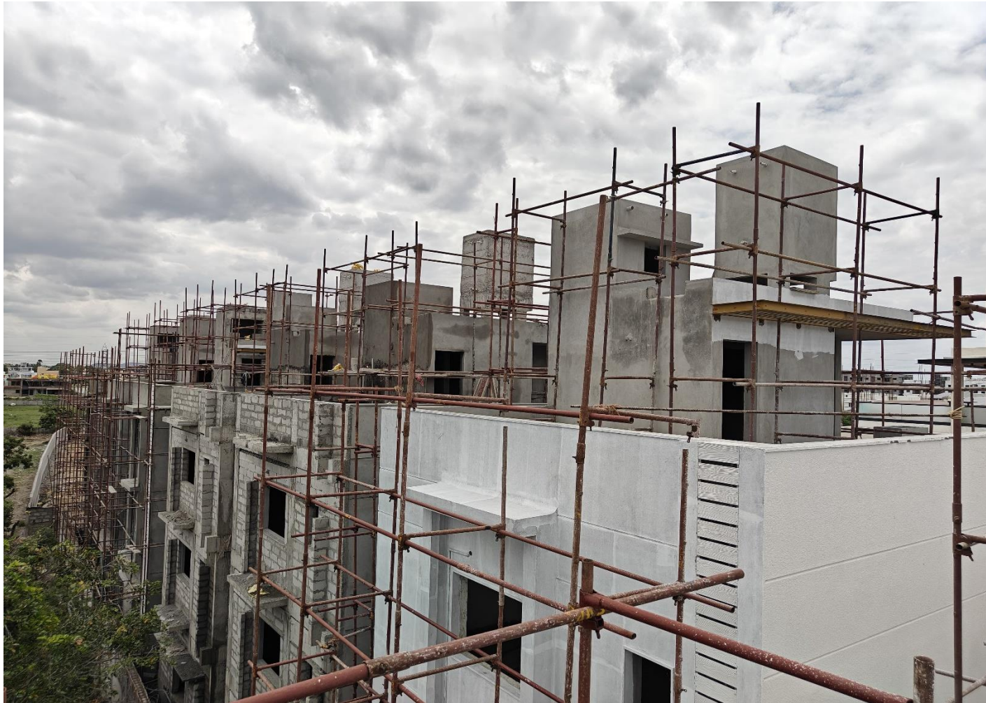
Villa No 6 – 11 headroom area plastering work in progress
