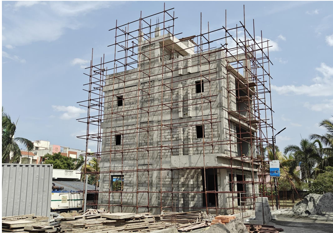
Villa No 3- External Scaffolding fixing work in progress
