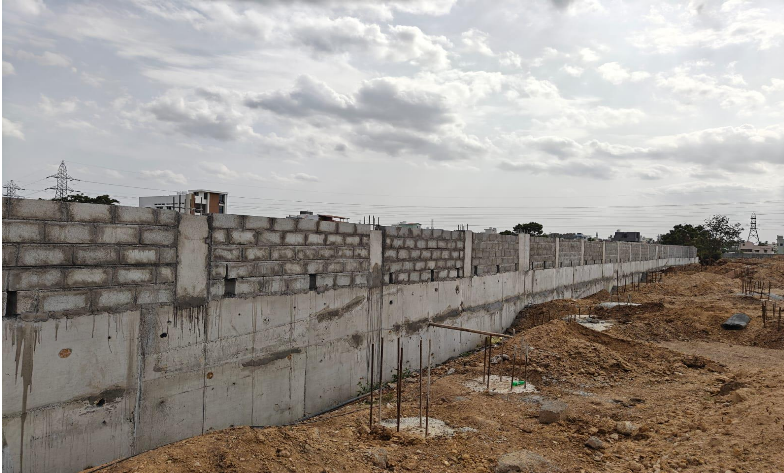
South Side Compound wall blockwork in progress
