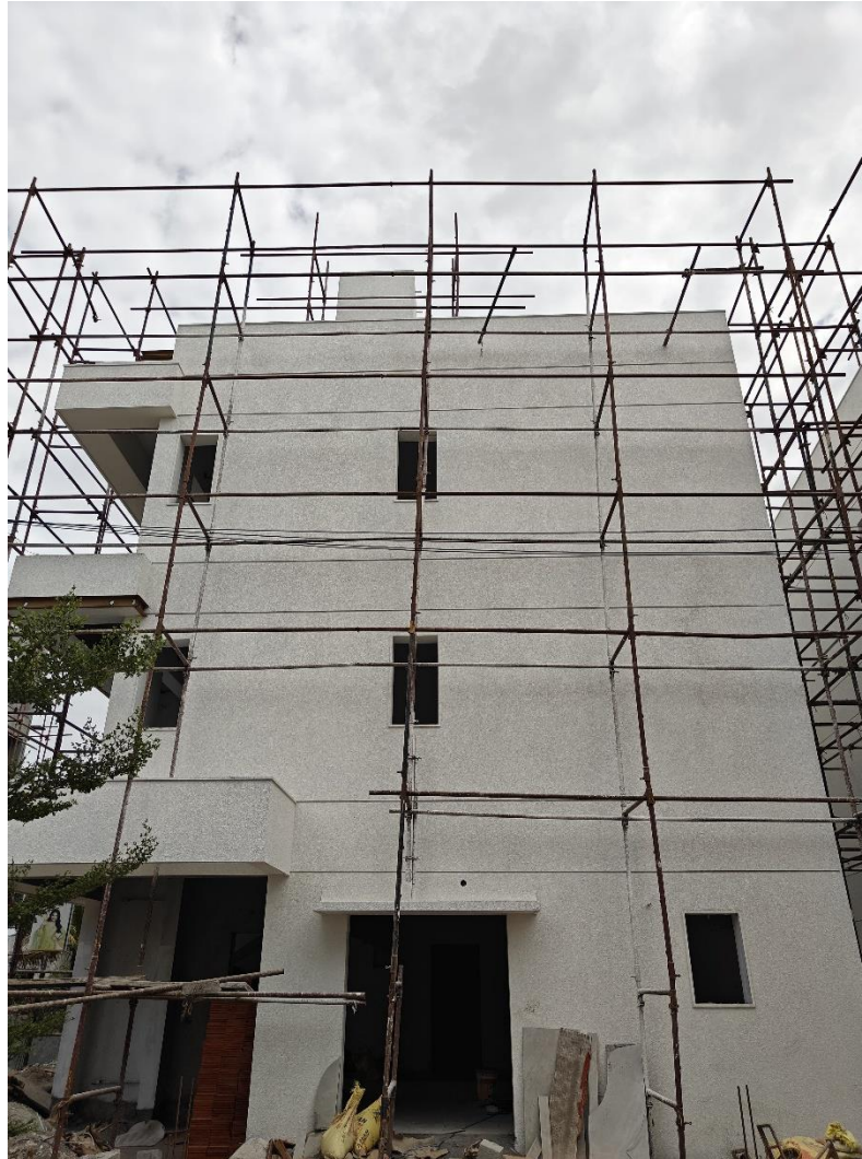
Villa No 5 – North side external wall pebble texture applying work in progress
