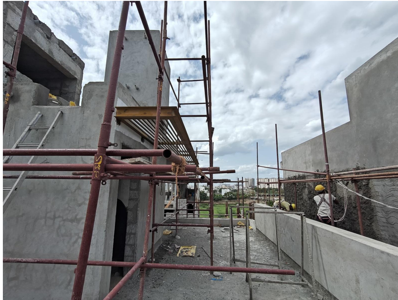
Villa No 9 – Terrace area MS Percola fixing work in progress
