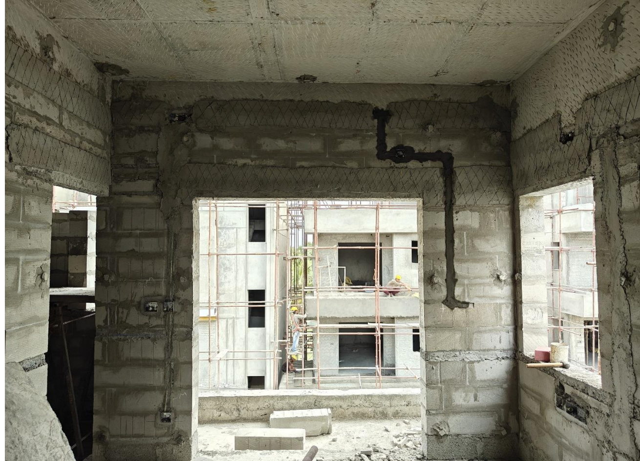
Villa No 13– SF Bedroom Electrical pipeline laying work in progress
