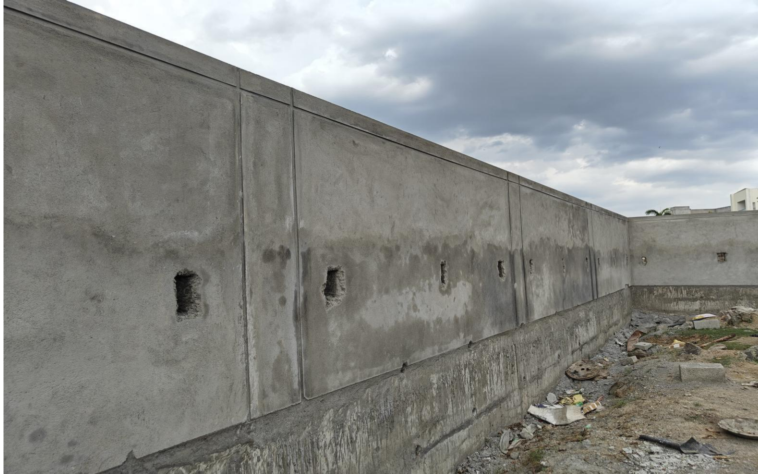
North Side Compound wall internal plastering work in progress
