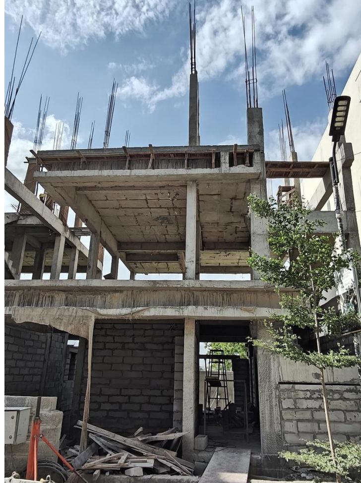
Villa No 15– SF Column concreting work completed
