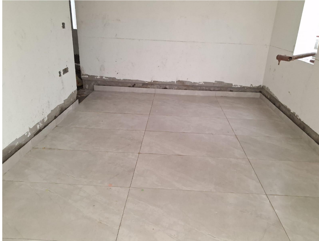
Villa No 5 – FF Bedroom Flooring tile laying work in progress
