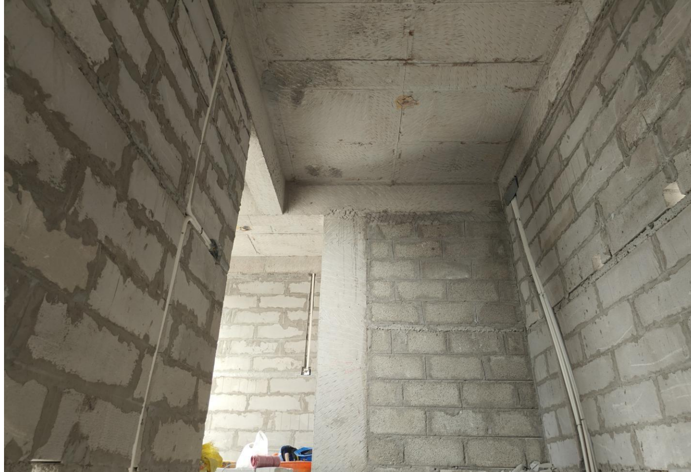
Villa No 7- Headroom Electrical pipeline laying work in progress
