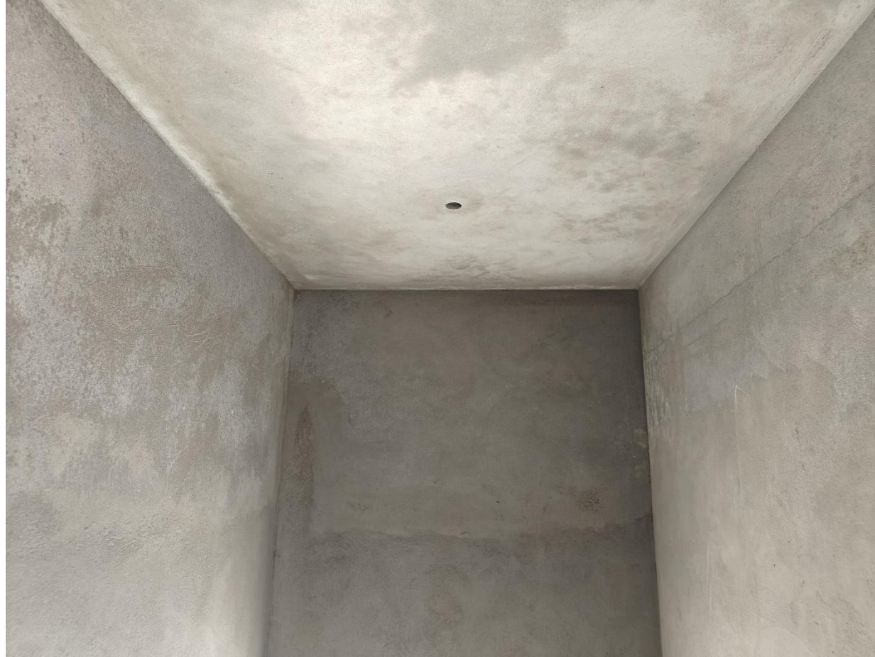
Villa No 7- FF Bedroom Internal plastering work in progress
