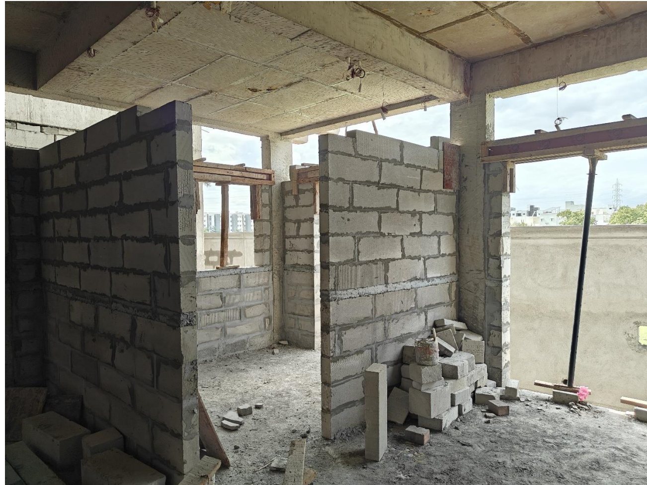
Villa No 14– Ground floor blockwork in progress
