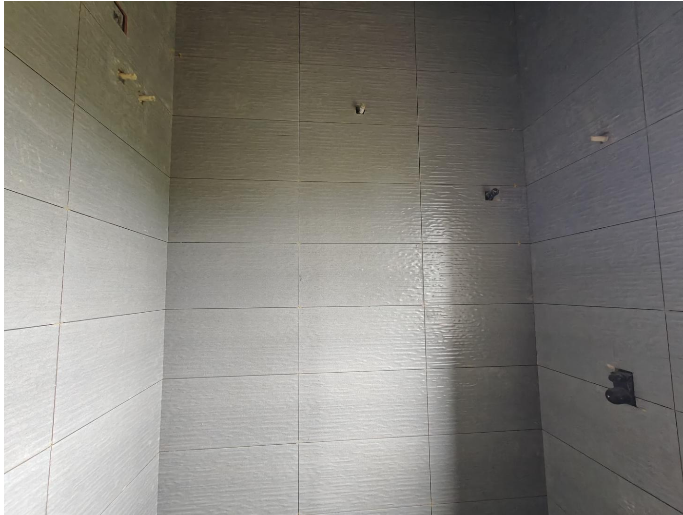
Villa No 9 – SF bedroom toilet wall tile laying work in progress
