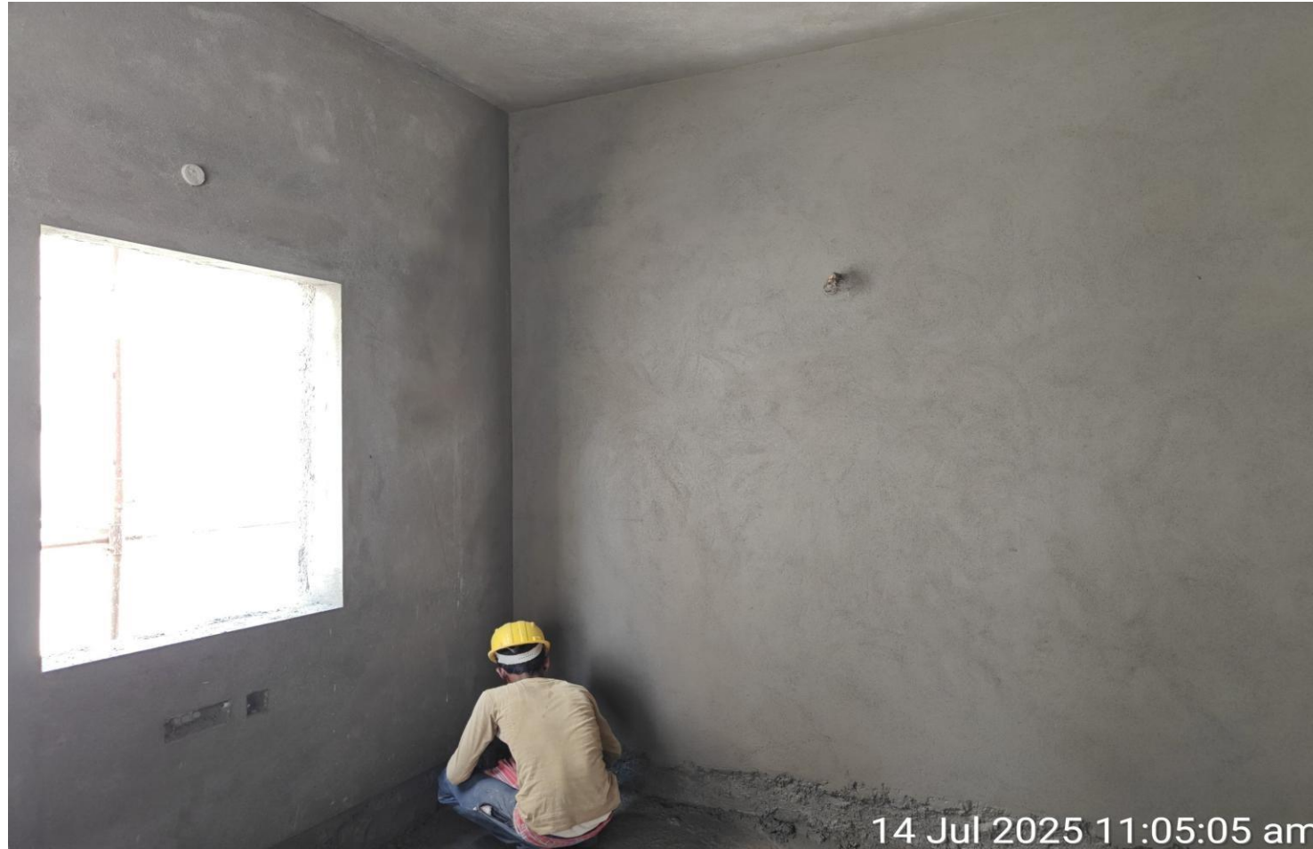
Villa No 13– FF Bedroom internal plastering work in progress
