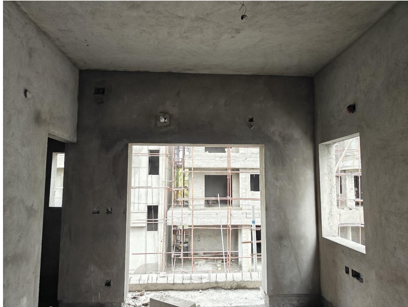
Villa No 13– FF Bedroom internal plastering work in progress
