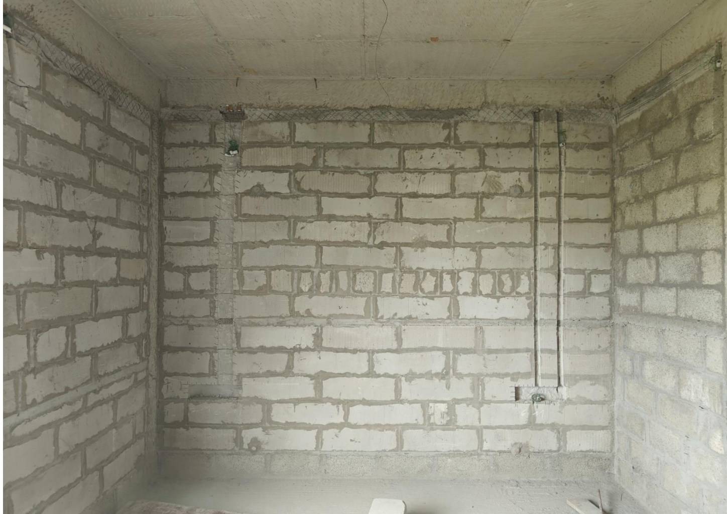
Villa No 7- SF Electrical pipeline wall chasing work in progress
