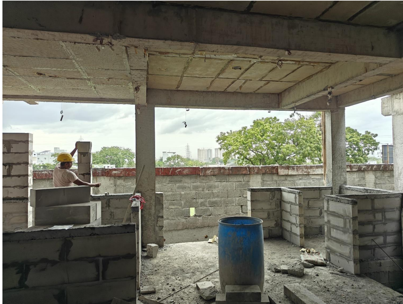
Villa No 14– Ground floor blockwork in progress
