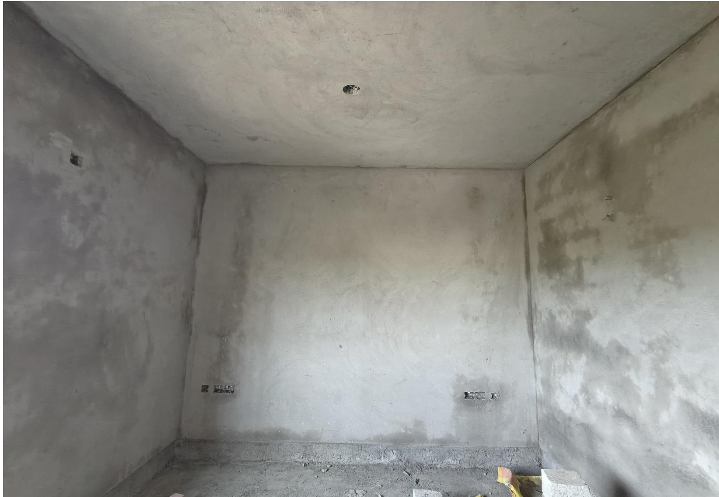
Villa No 10- FF Bedroom internal plastering work in progress
