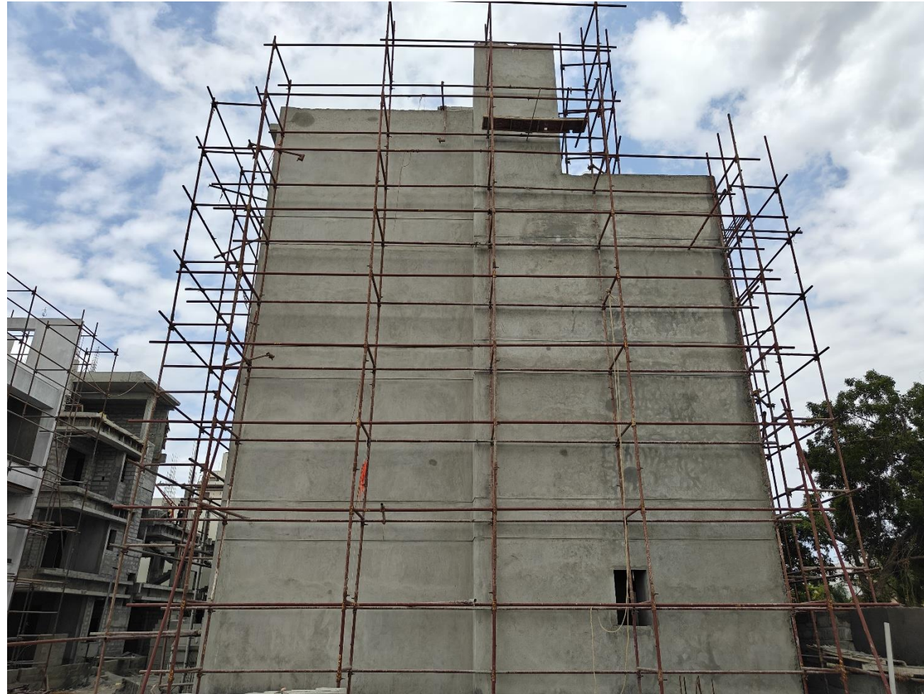
Villa No 11- Westside external plastering work in progress
