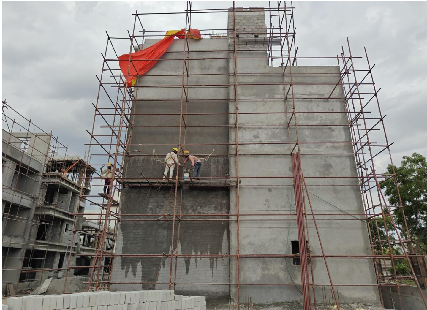
Villa No 11- Westsideexternal plastering work in progress
