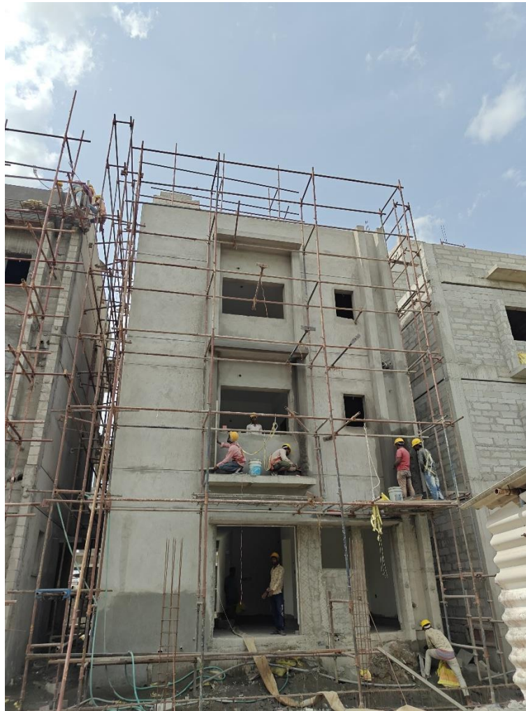
Villa No 9 – Southside external plastering work in progress
