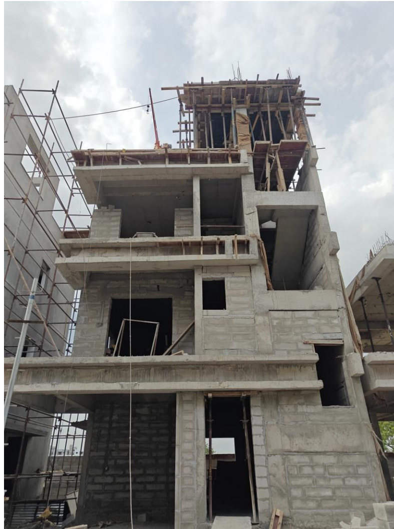
Villa No 13 – Head room Roof slab concreting work completed
