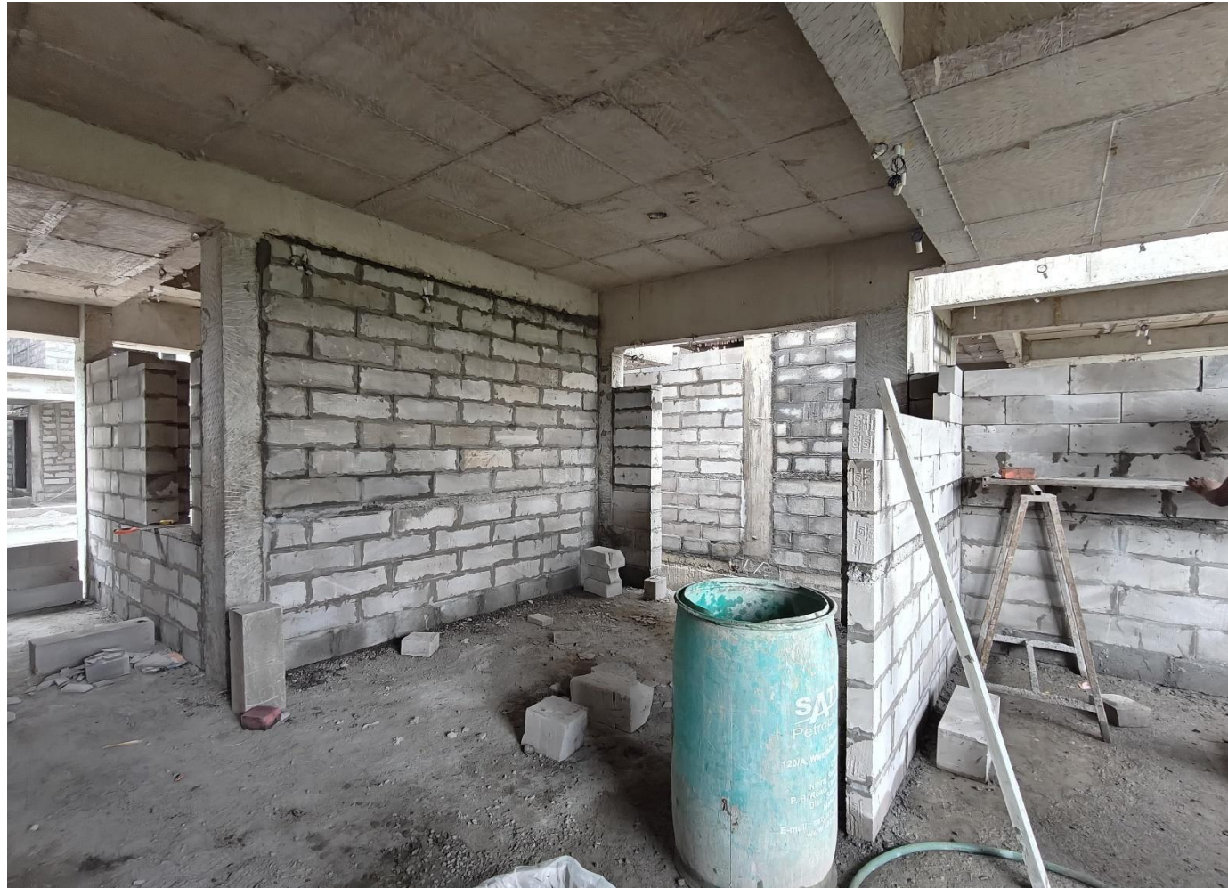
Villa No 15– Ground floor blockwork in progress
