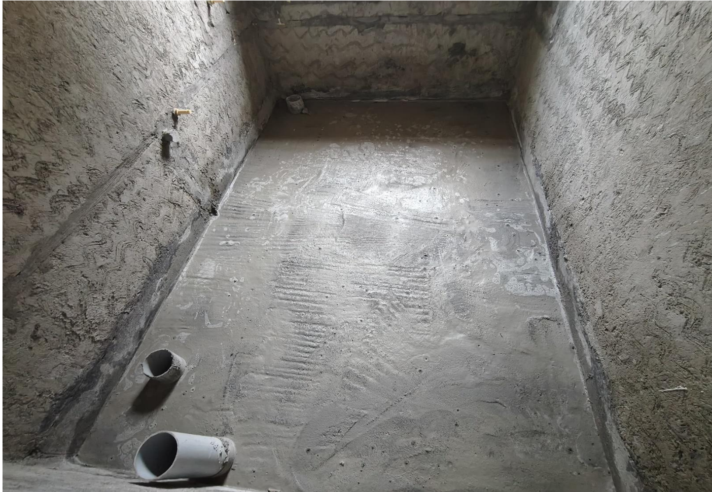
Villa No 12 – FF Toilet Sunken screed concreting work in progress
