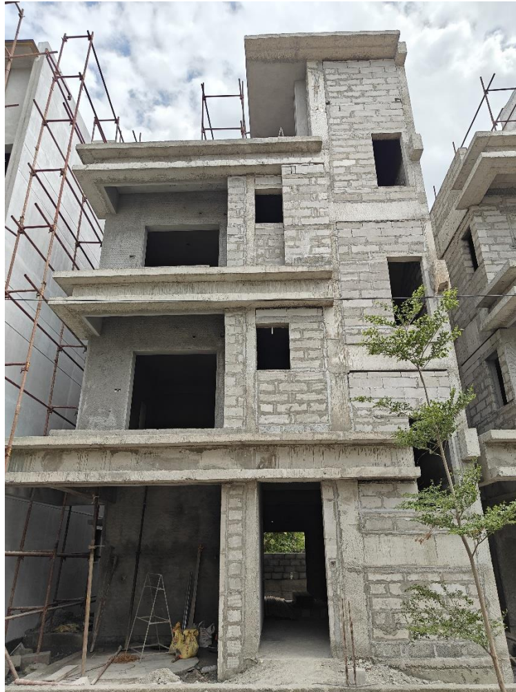
Villa No 7- FrontElevationview
