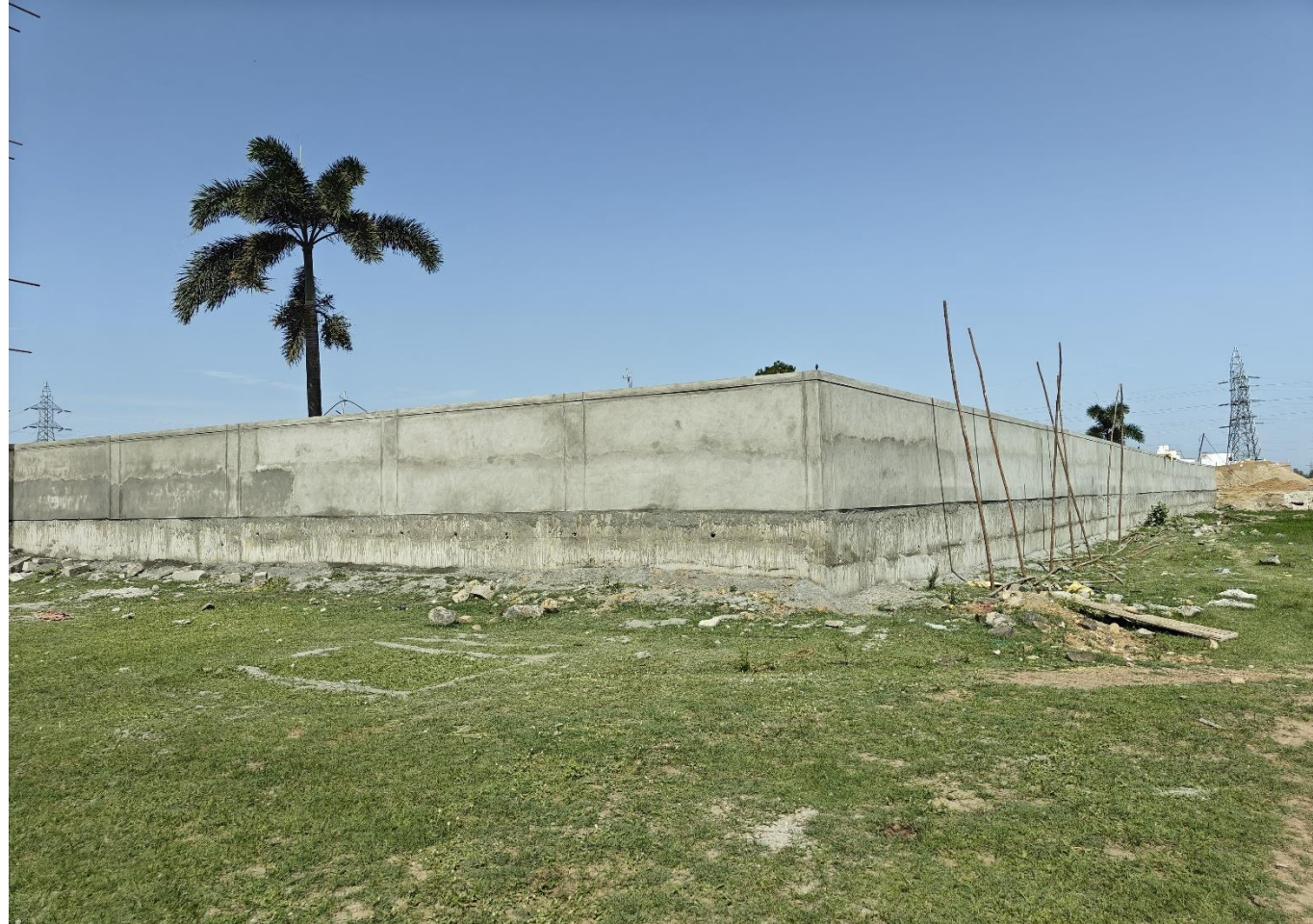
Phase 1 - Northside compound wall external plastering work in progress
