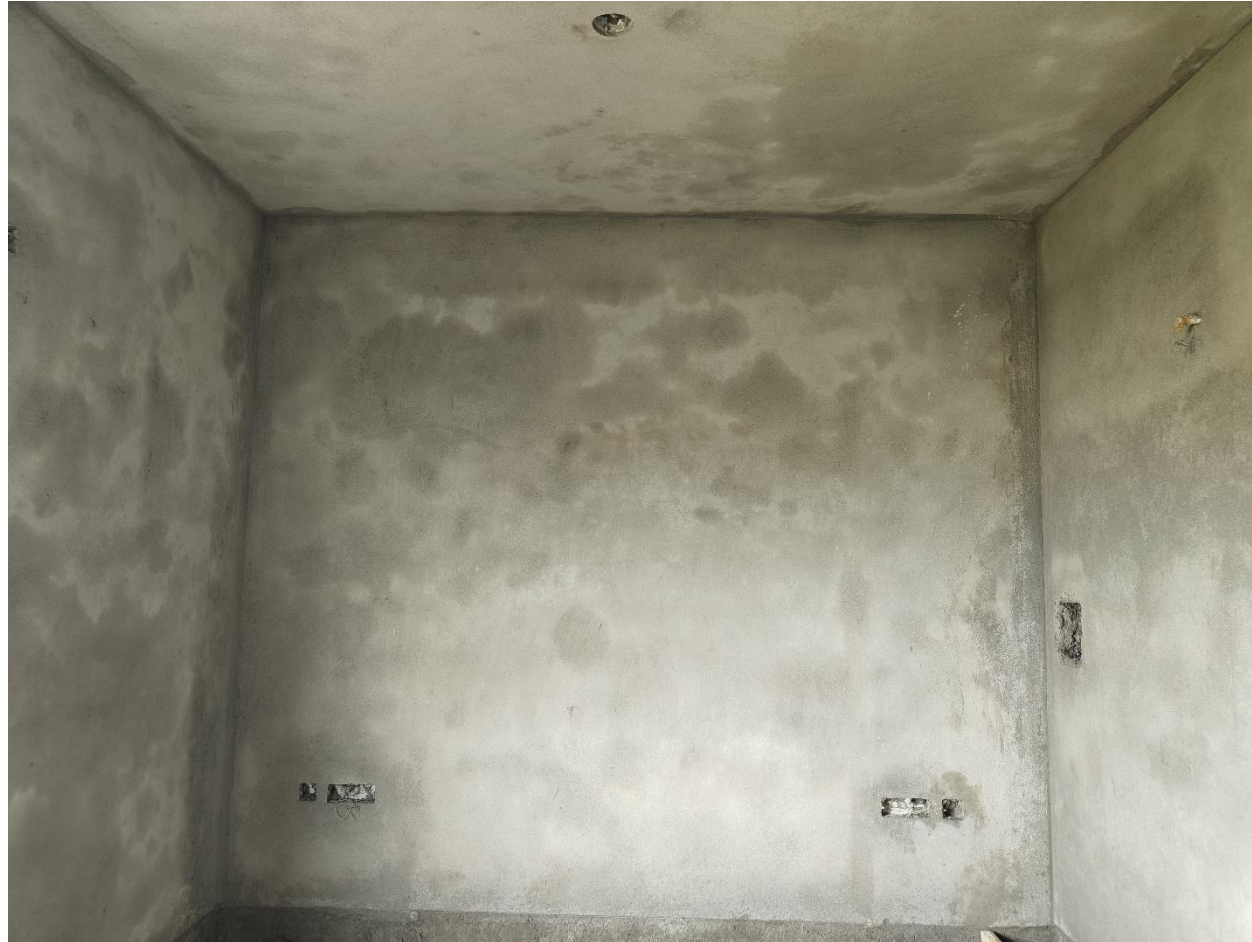
Villa No 8 - FF bedroom internal plastering work in progress
