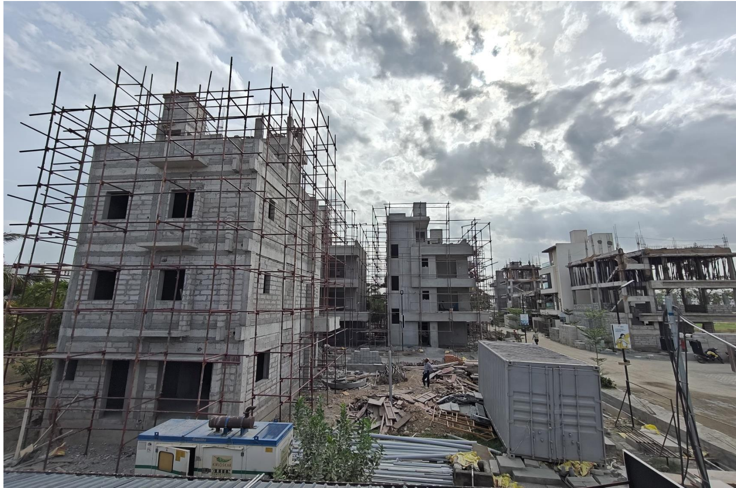
Villa No 3- External Scaffolding fixing work in progress
