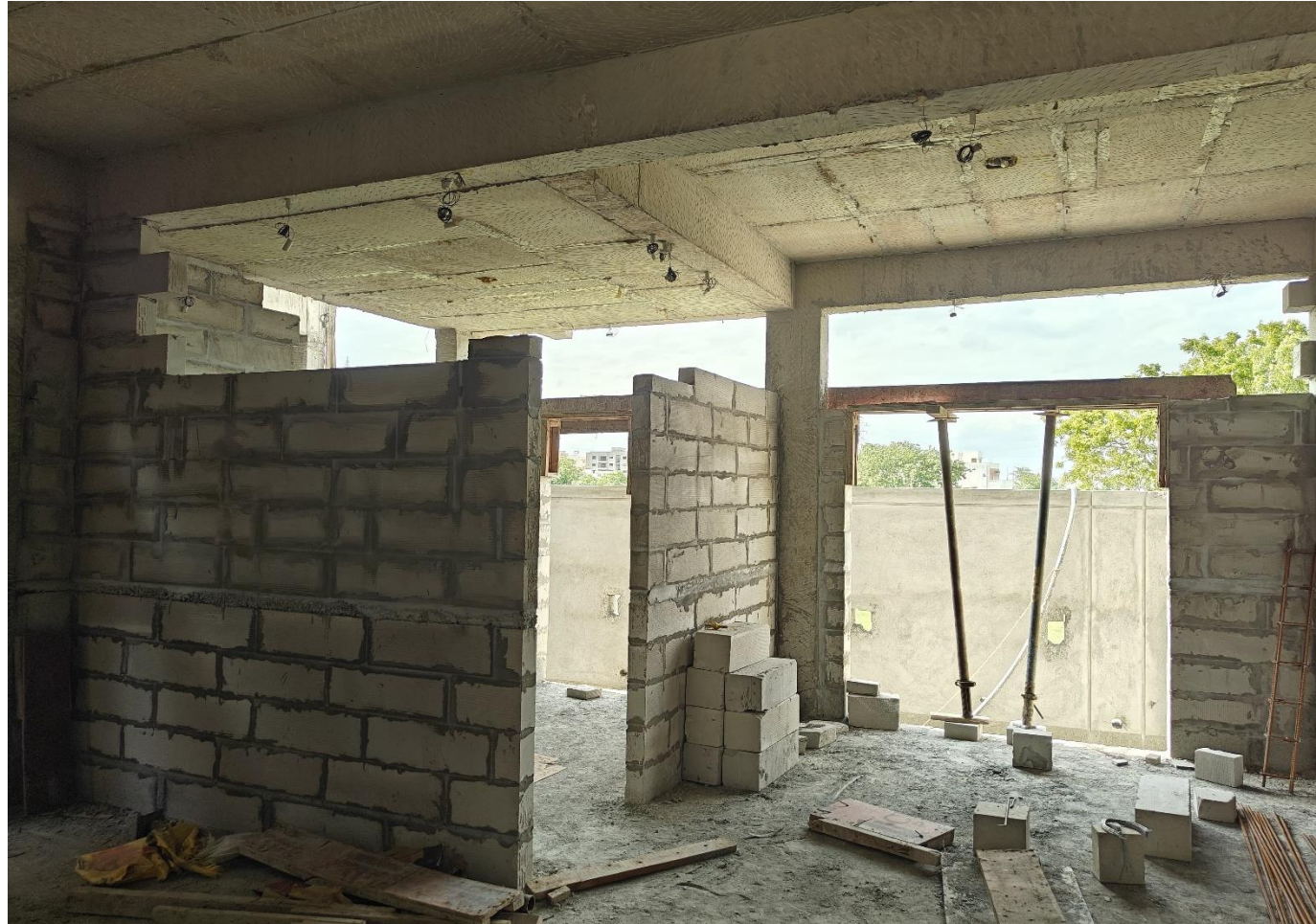
Villa No 15– Ground floor blockwork in progress
