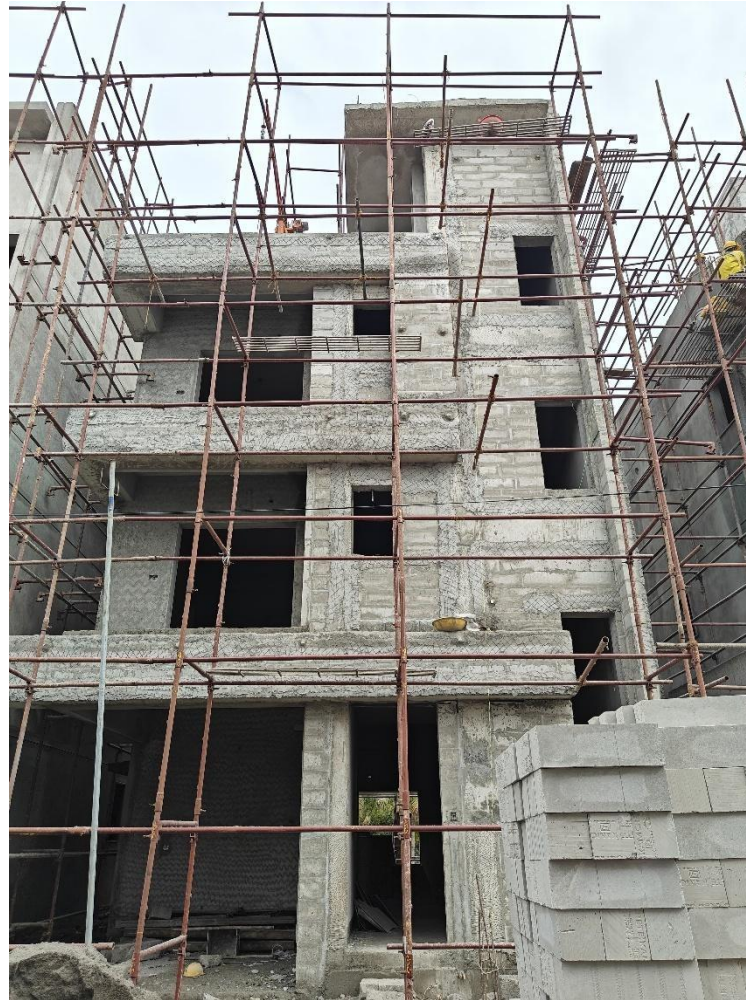
VillaNo 10- Front elevation plastering preparation work in progress
