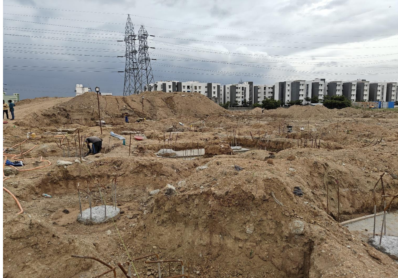
Phase 2 – villa no 46 - pile cap preparation work in progress
