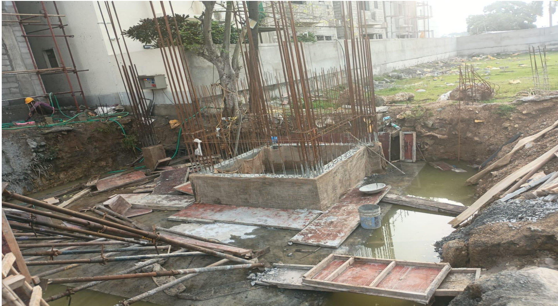
Villa No-18&19 Club House Lift Pedestal Column Concrete Completed
