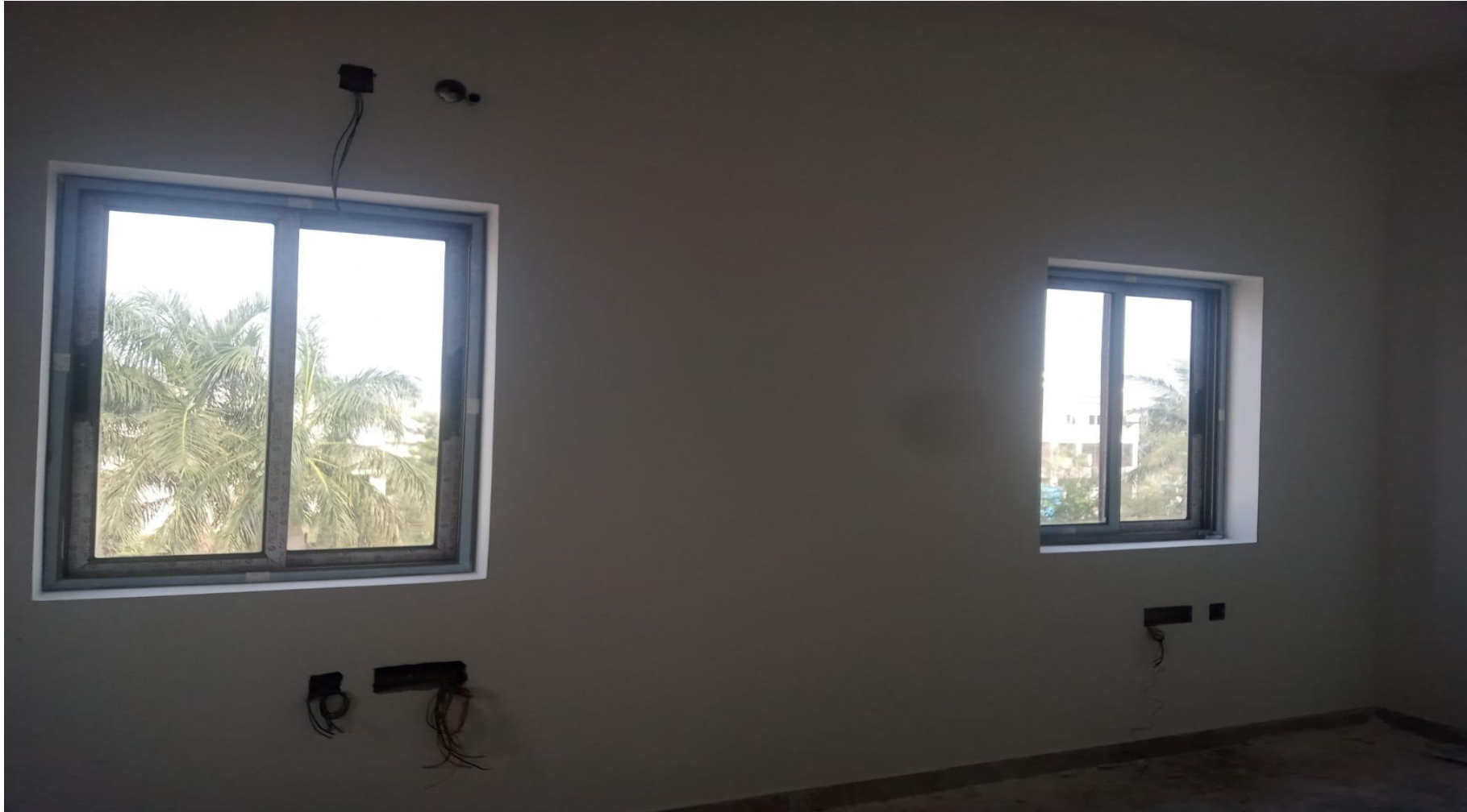
Villa No 3 Wire Rope Pulling Work In Progress
