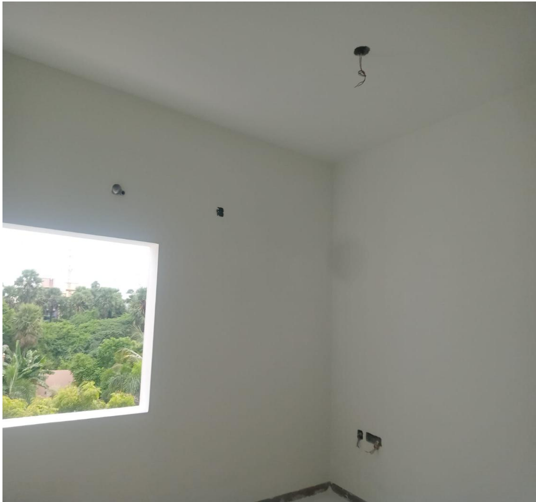
Villa No 6- Putty Scrapping Work On Progress
