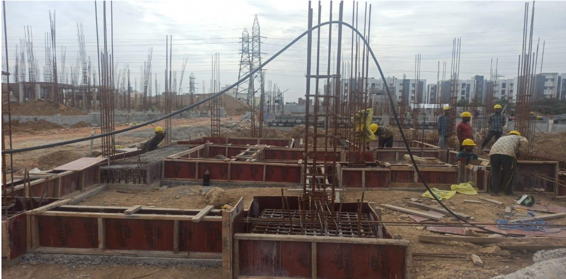
Phase 2 – villa no 71 Plinth Beam Shuttering Work In Progress
