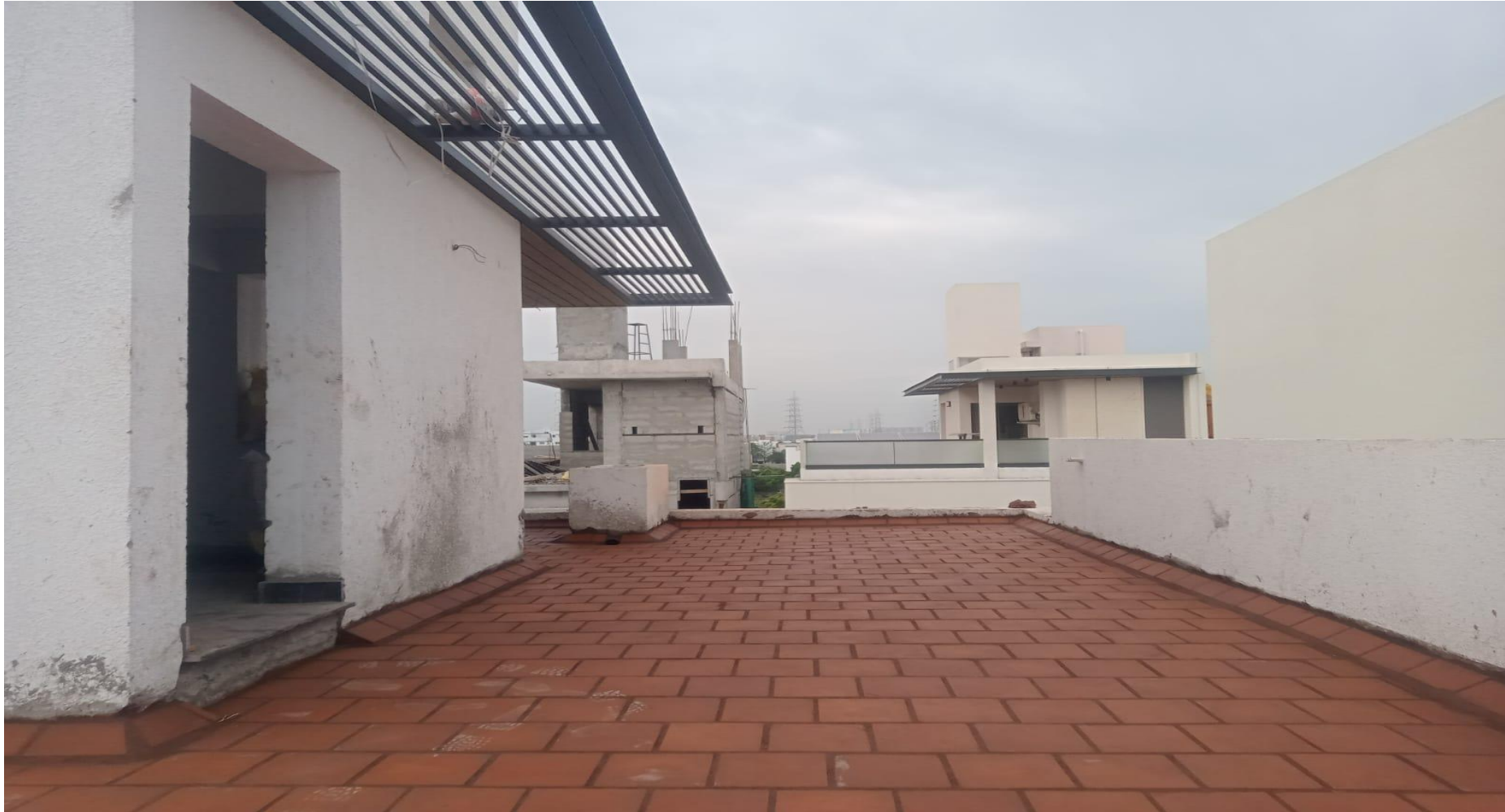
Villa No 7-Terrace Area Clay Tiles Laying Completed
