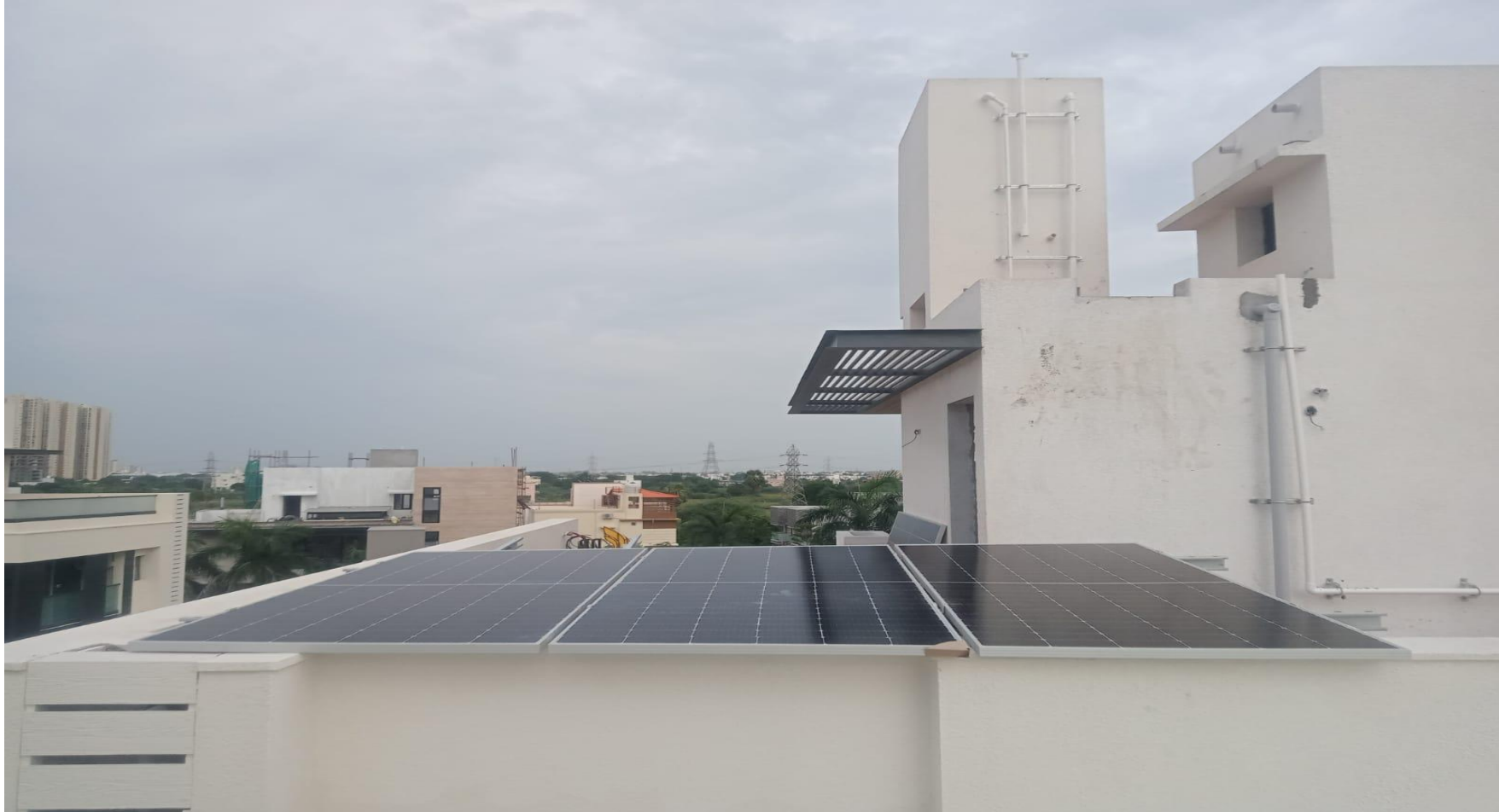
Villa No - 5 Solar Panel Fixing Work On Progress
