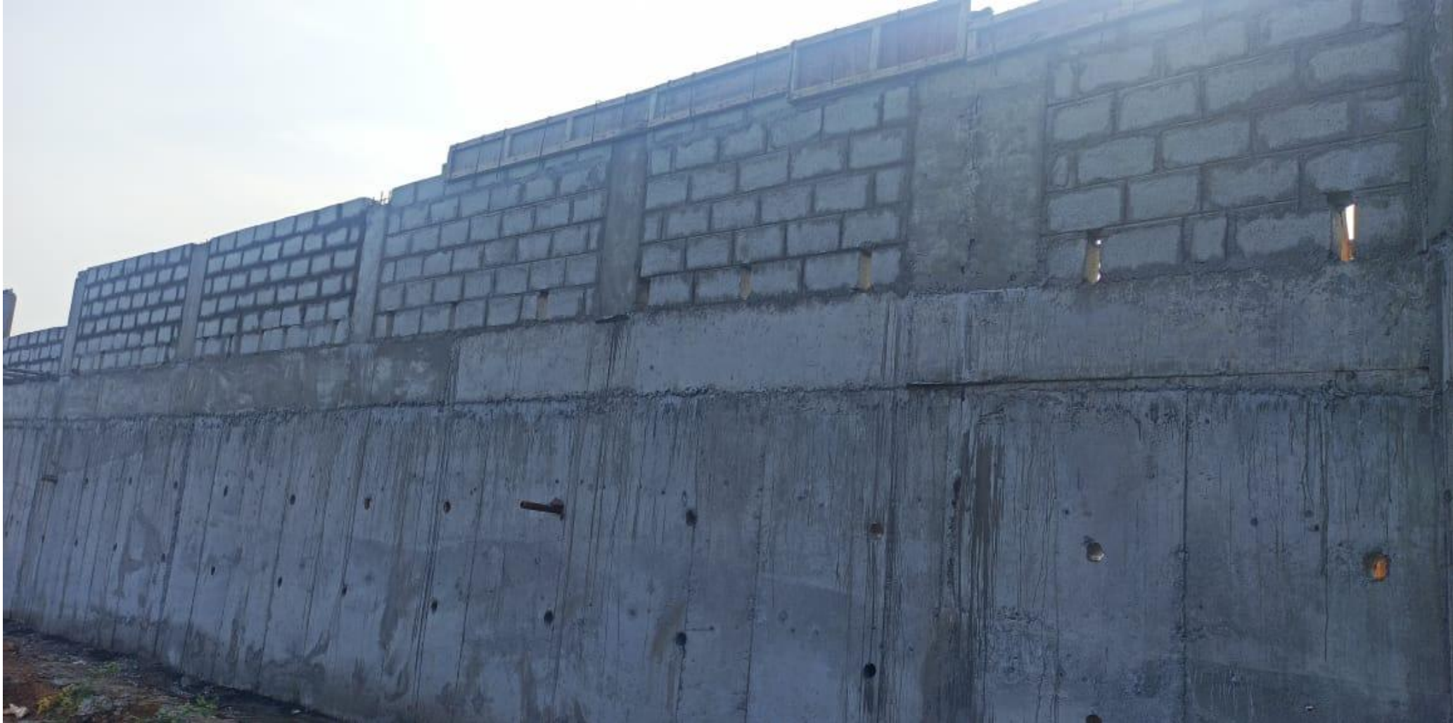
Phase 2 Compound Wall Block Work On Progress
