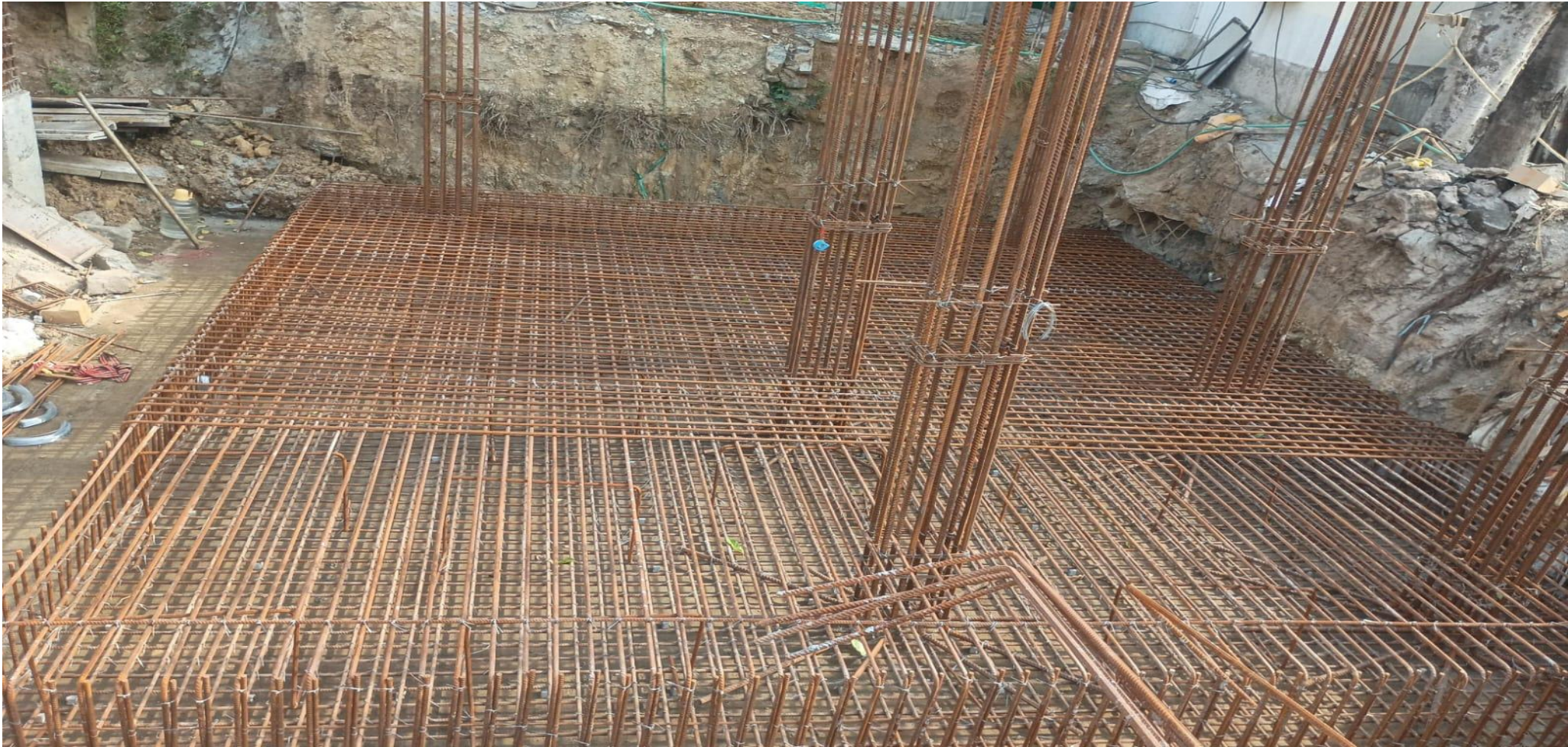
Villa No-18&19 Club House Footing Reinforcement Working Progress
