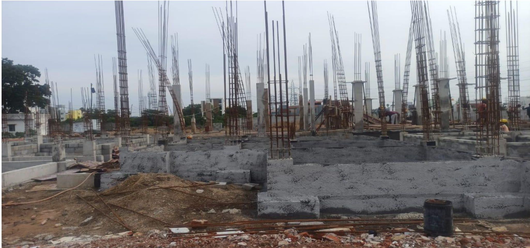
Phase 2 – villa no 56 DPC Work Completed
