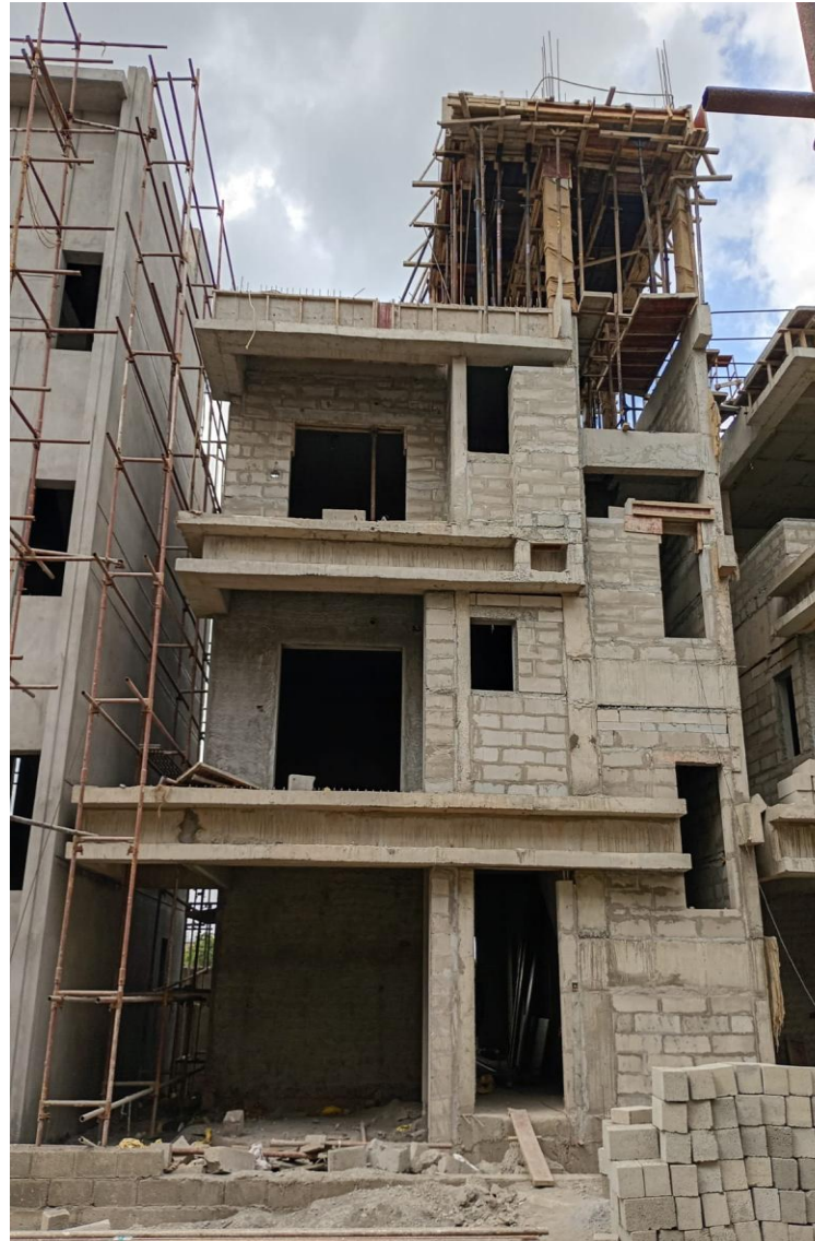
Villa No 14 – Front Elevation Head Room Concrete Pouring Completed
