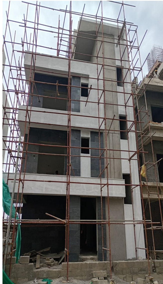
Villa No 13- Front Elevation Primer work in Progress
