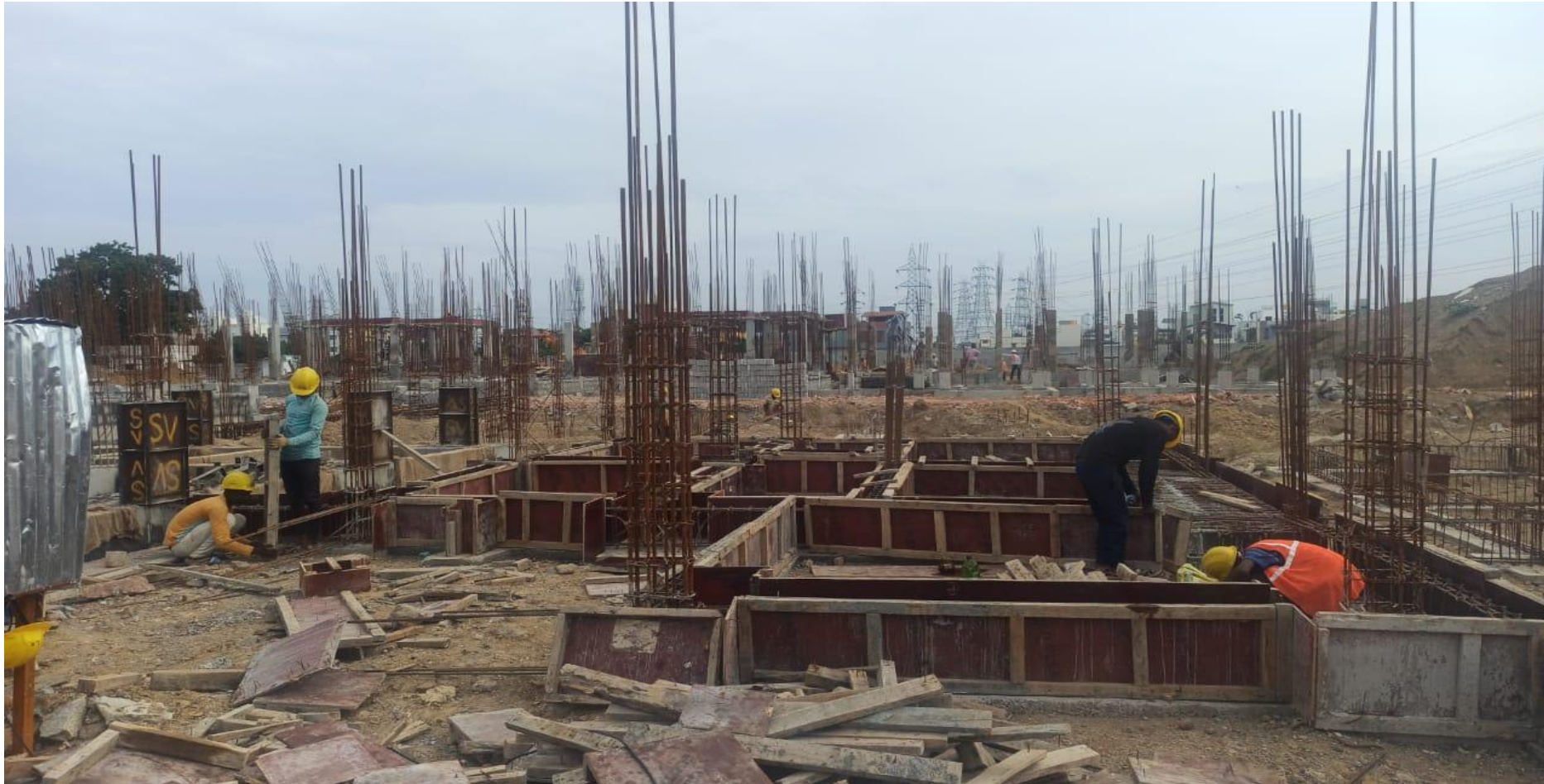
Phase 2 – villa no 78 Plinth Beam Shuttering Work In Progress
