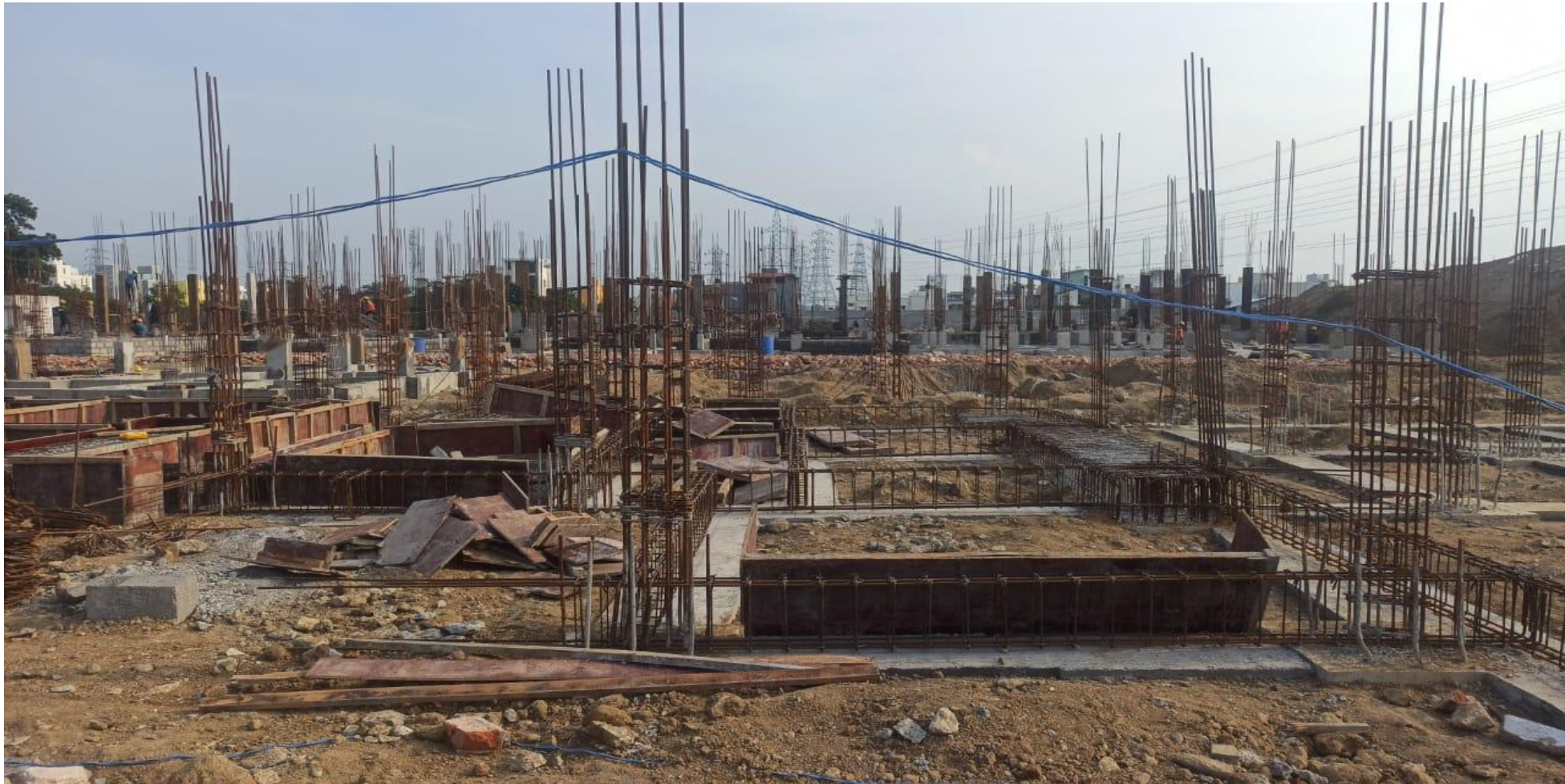
Phase 2 – villa no 77 Plinth Beam Reinforcement Work In Progress
