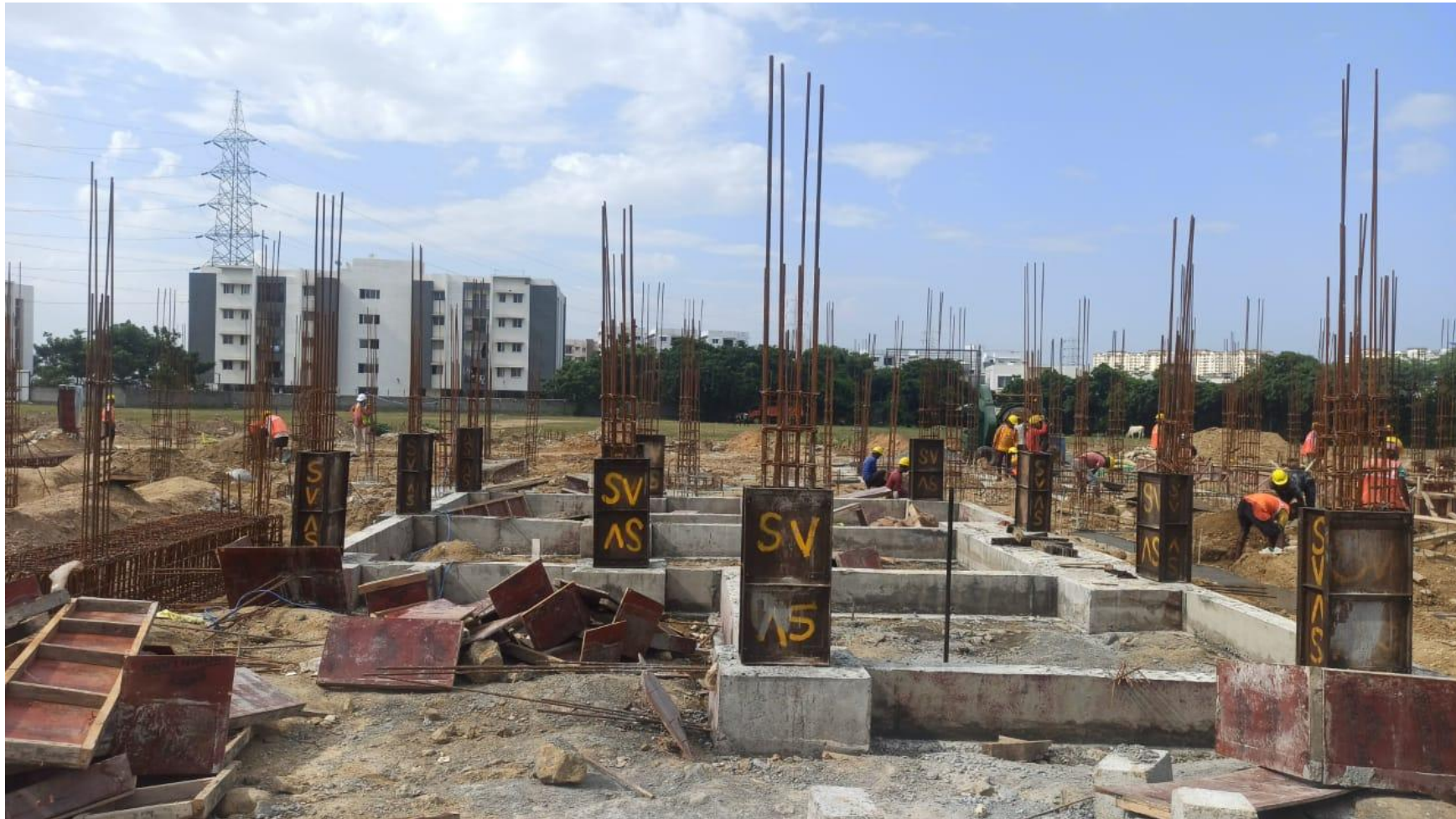
Phase 2 – villa no 68 Pedestal Column Shuttering Work Progress
