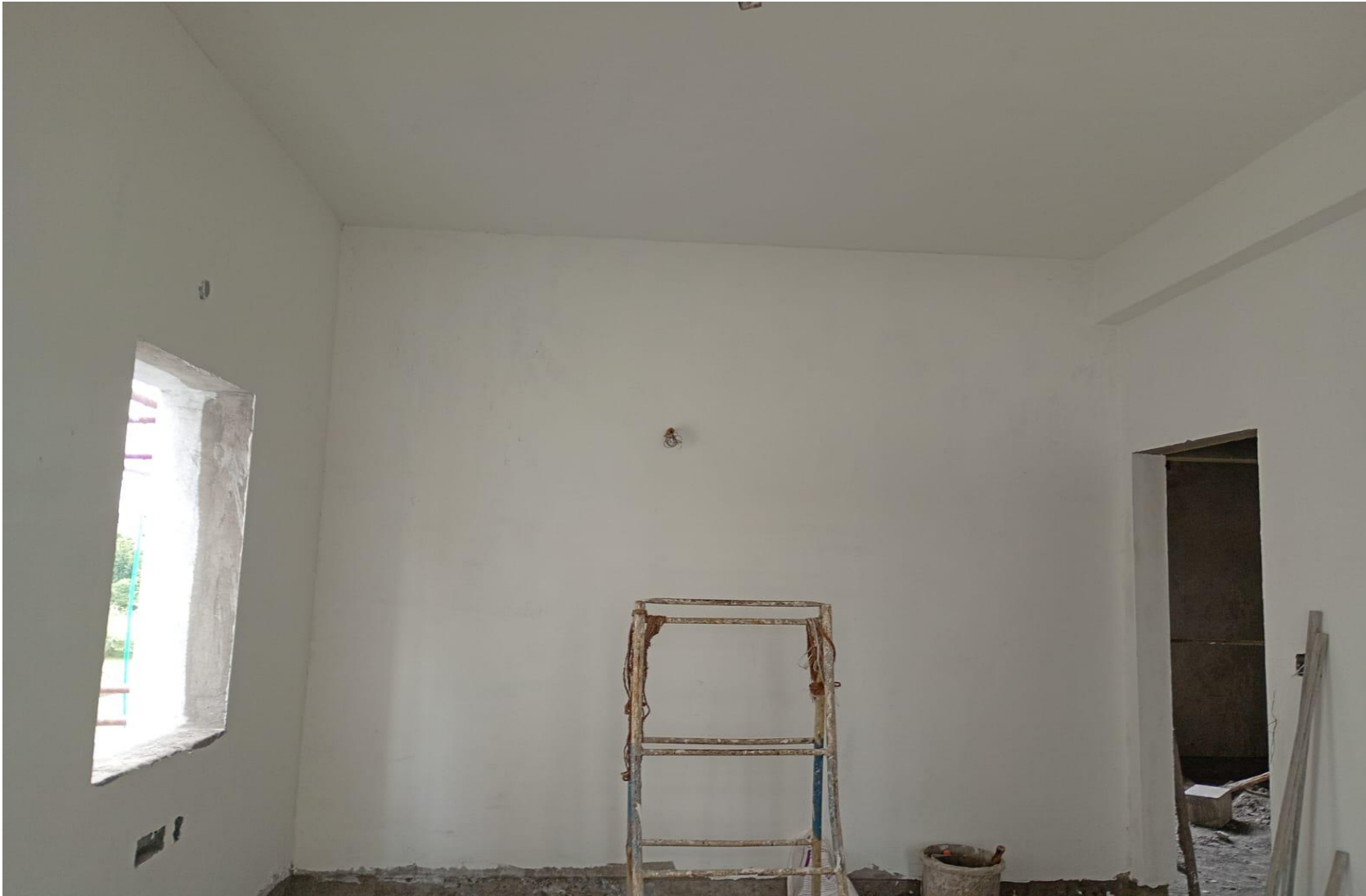
Villa No 13- FF &SF Wall 1st Coat Putty Work In Progress
