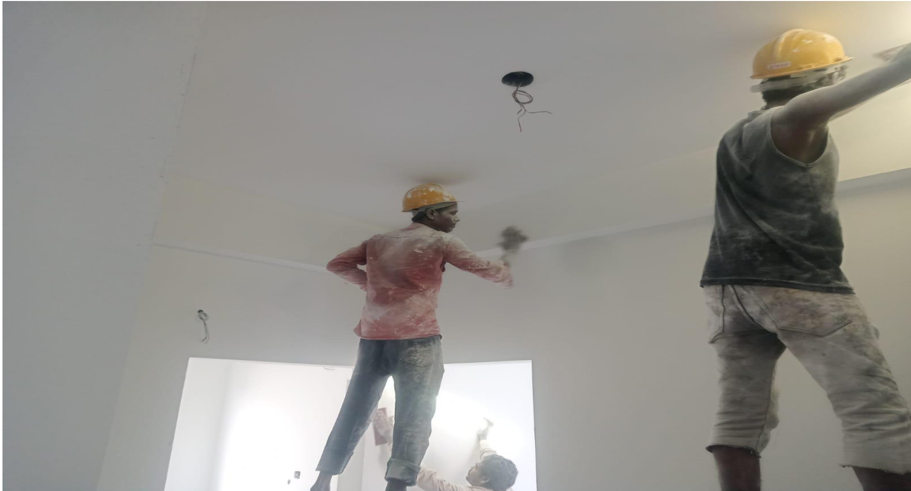
Villa No – 5 Putty Scraping Work In Progress
