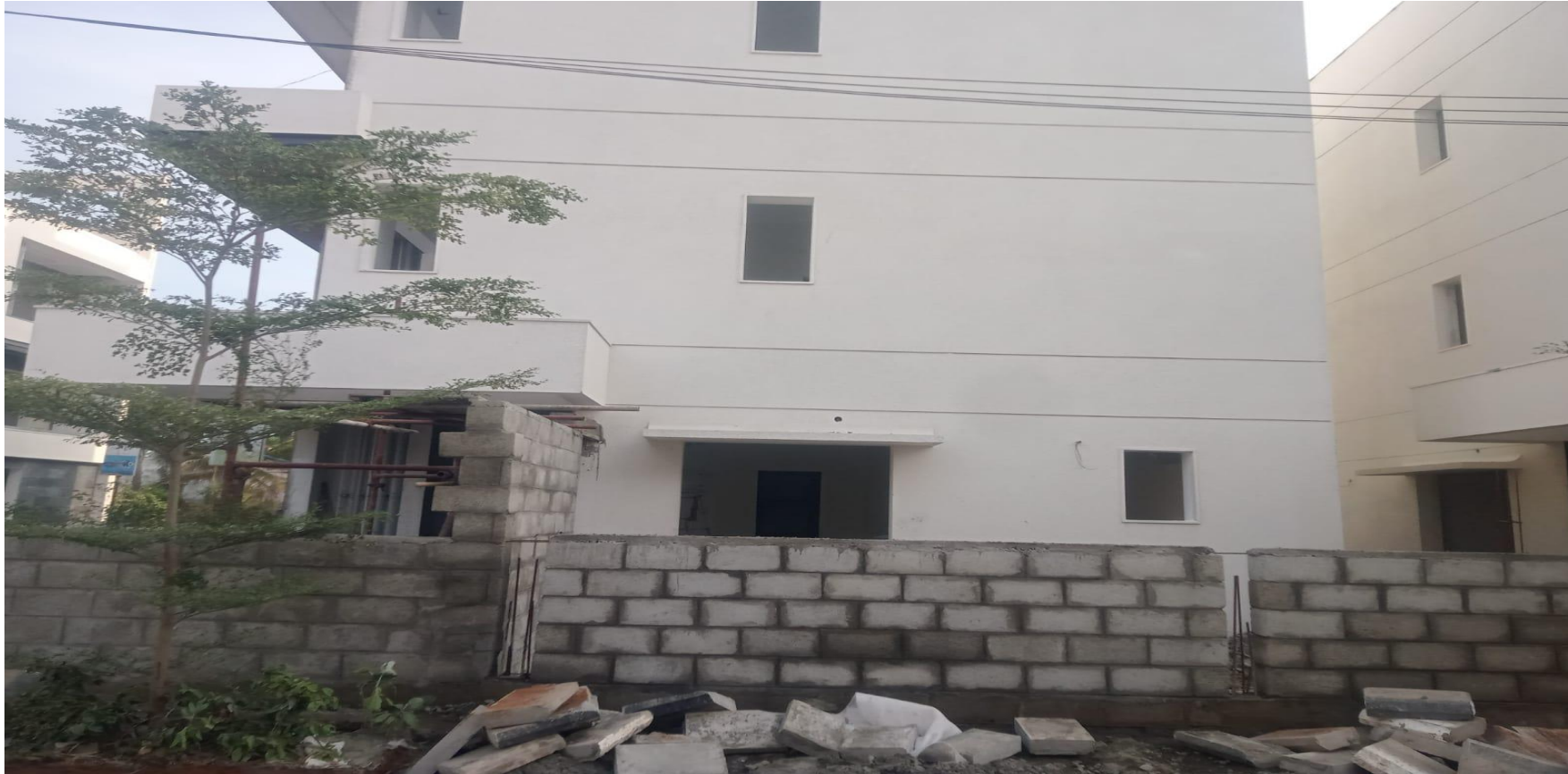
Villa No - 5 Compound Wall Block Work In Progress
