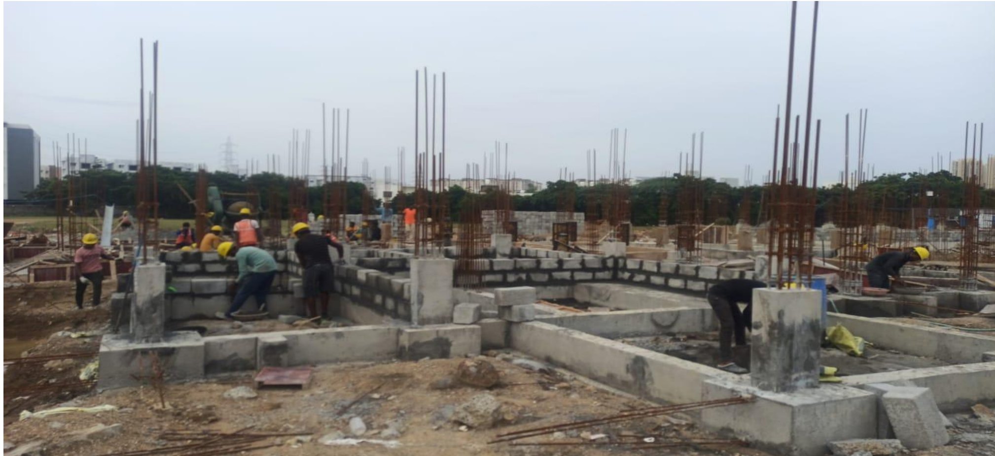
Phase 2 – villa no 68 Basement Block Work Progress
