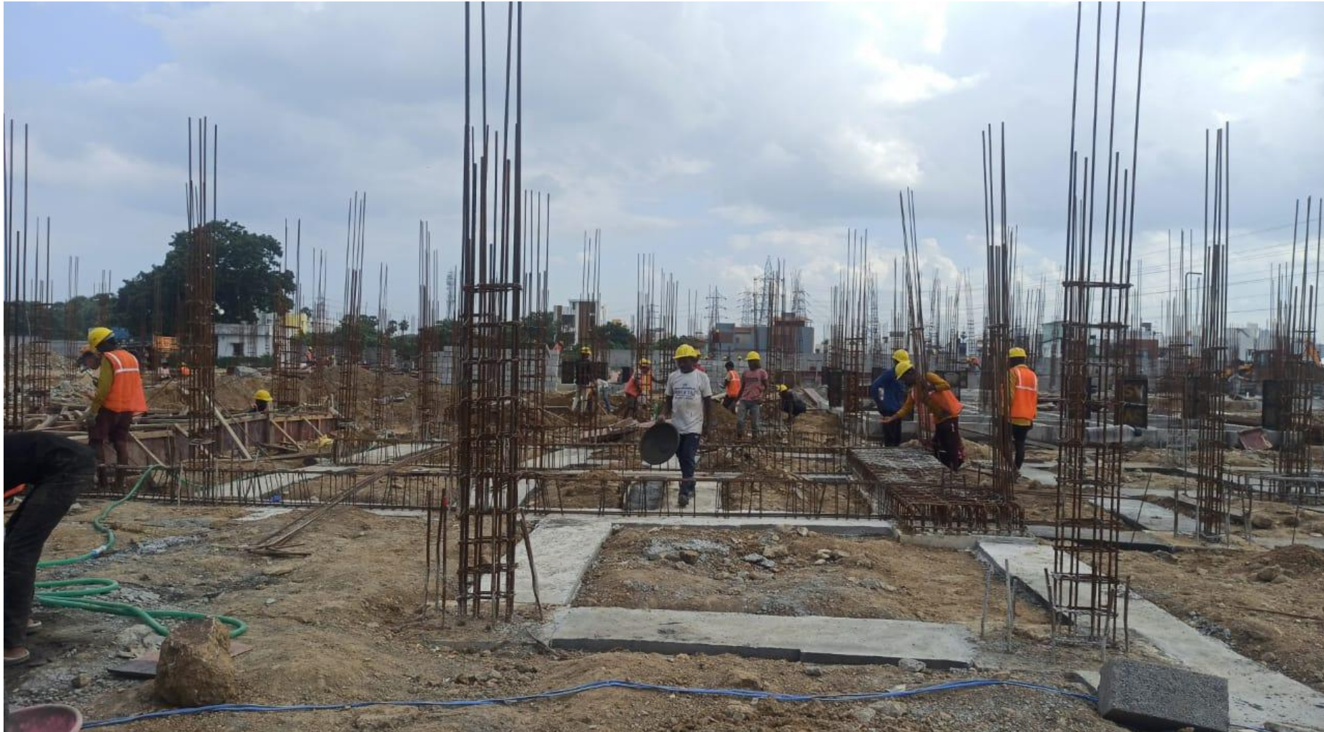
Phase 2 – villa no 75 Plinth Beam Reinforcement Work In Progress
