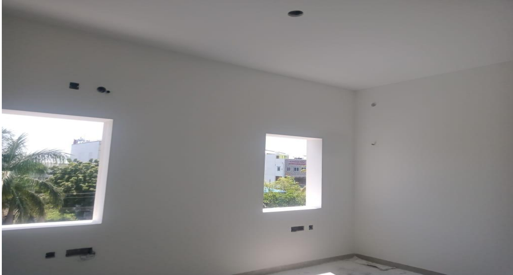
Villa No 3 FF 2 nd Coat Putty Work Completed
