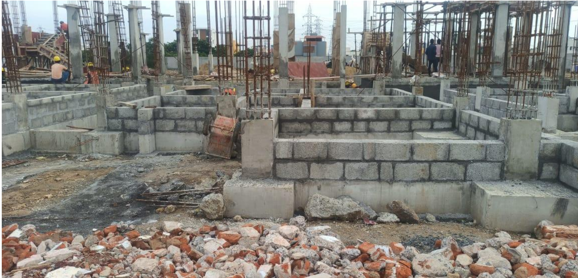
Phase 2 – villa no 58 Basement Block Work Completed
