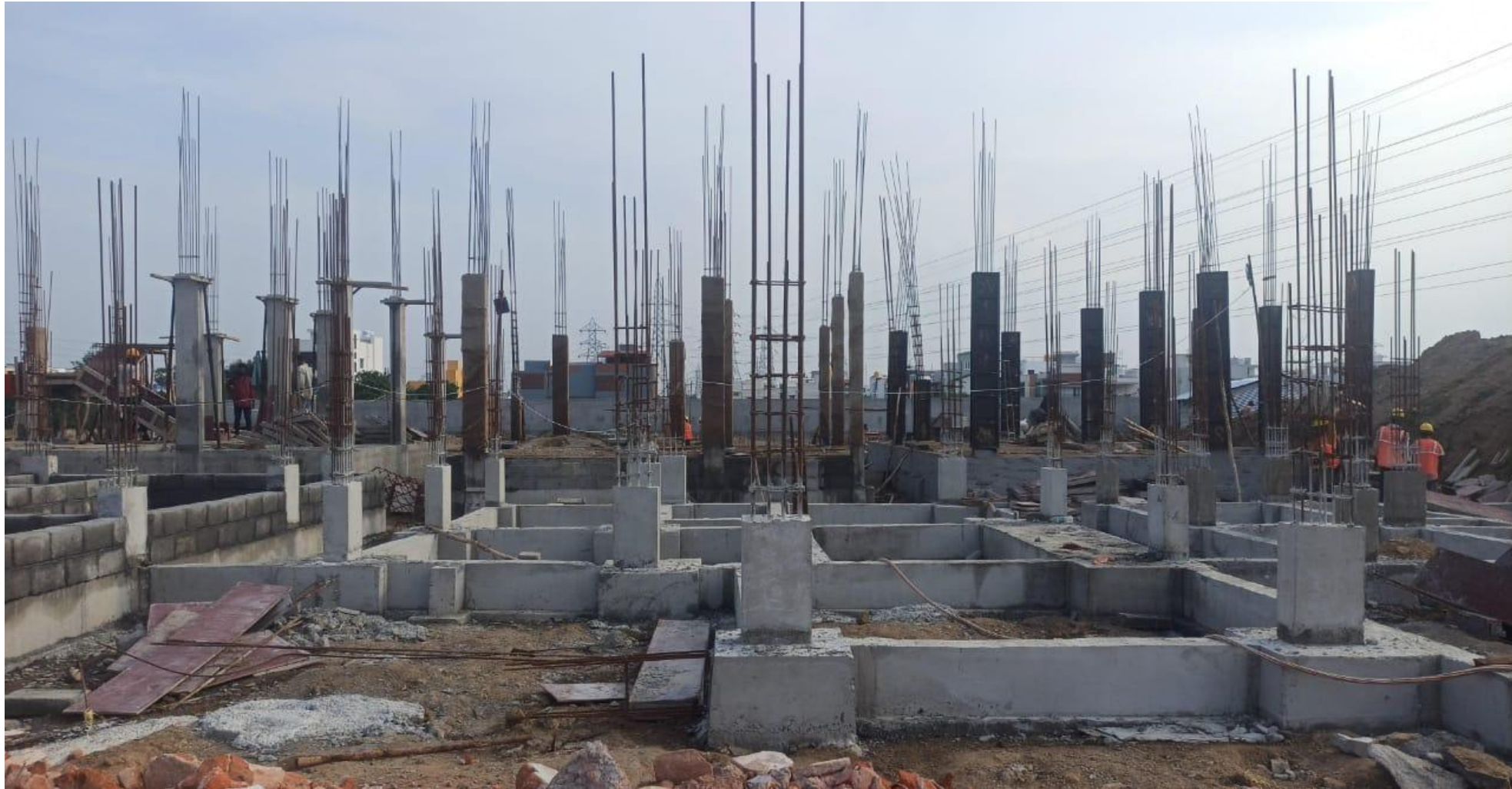
Phase 2 – villa no 60 Pedestal Column Concrete Completed
