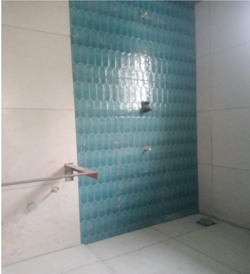
Villa No 8-FF&SF Toilets Tiles Laying Work In Progress
