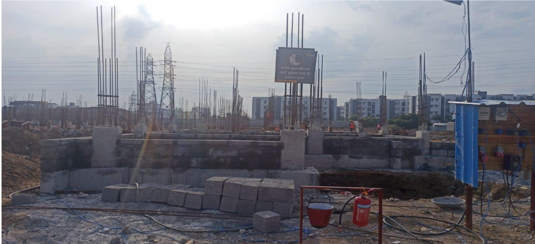
Phase 2 – villa no 73 Basement Block Work Completed
