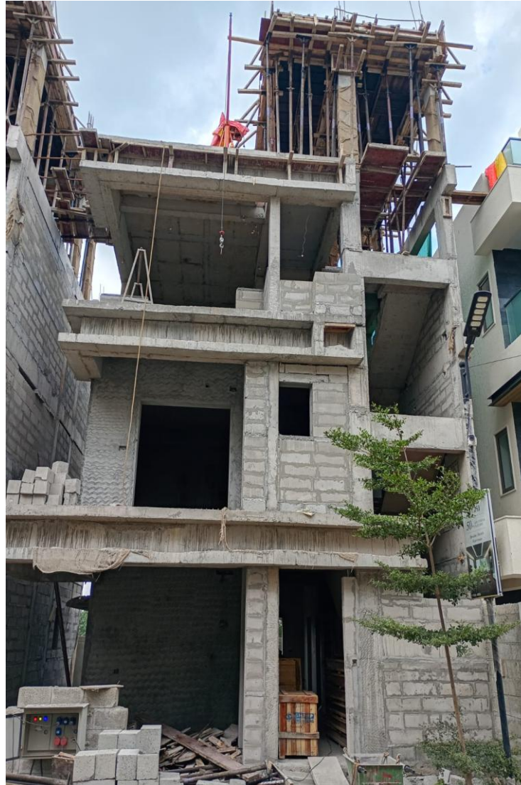
Villa No 15–Front Elevation Head Room Concrete Pouring Completed
