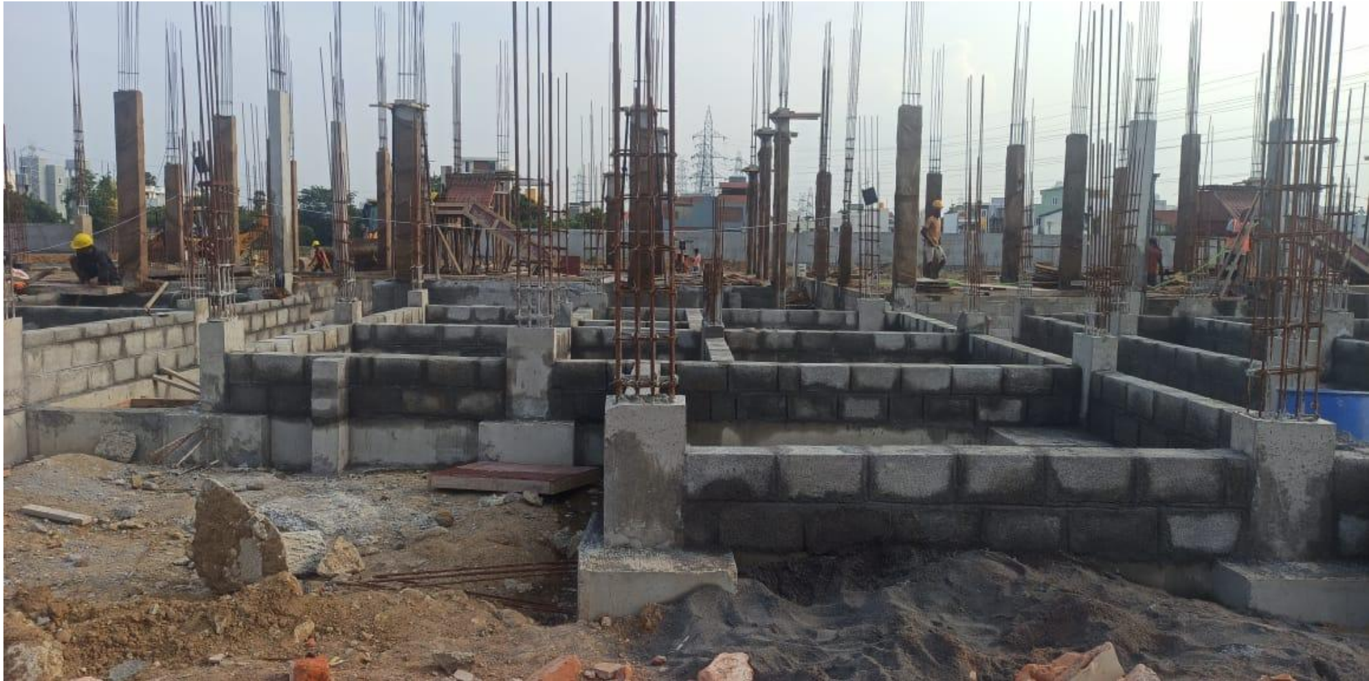
Phase 2 – villa no 57 Basement Block Work Completed
