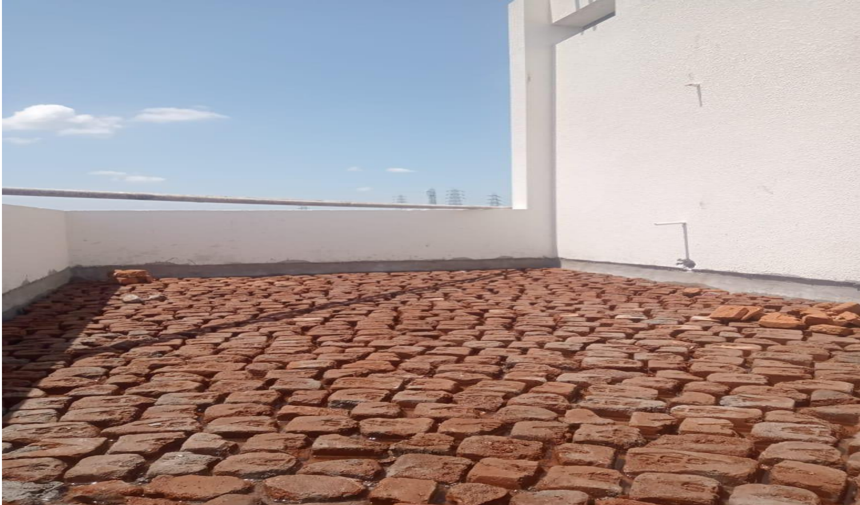
Villa No 3 Terrace Brick Bat Coba Laying Work In Progress
