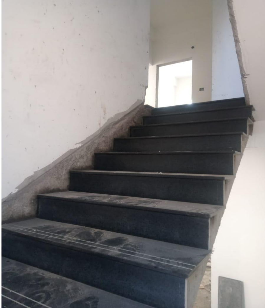
Villa No 7-Staircase Granite Laying Work Completed
