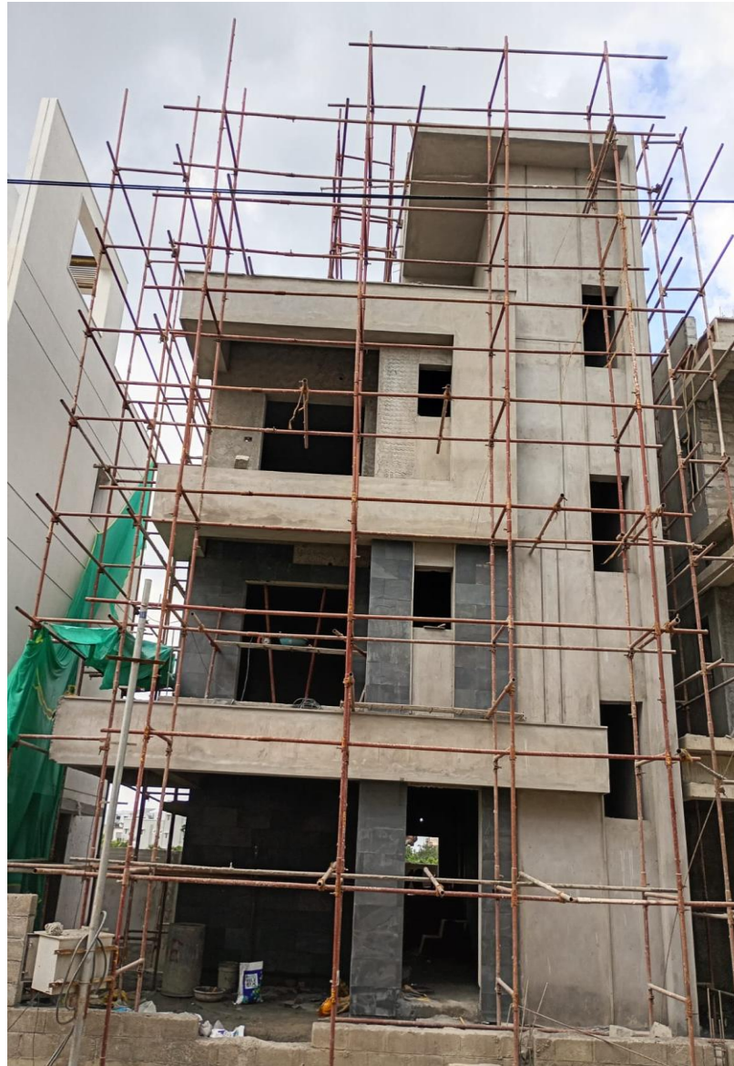
Villa No 13- Front Elevation Slate Tiles Laying Work In Progress
