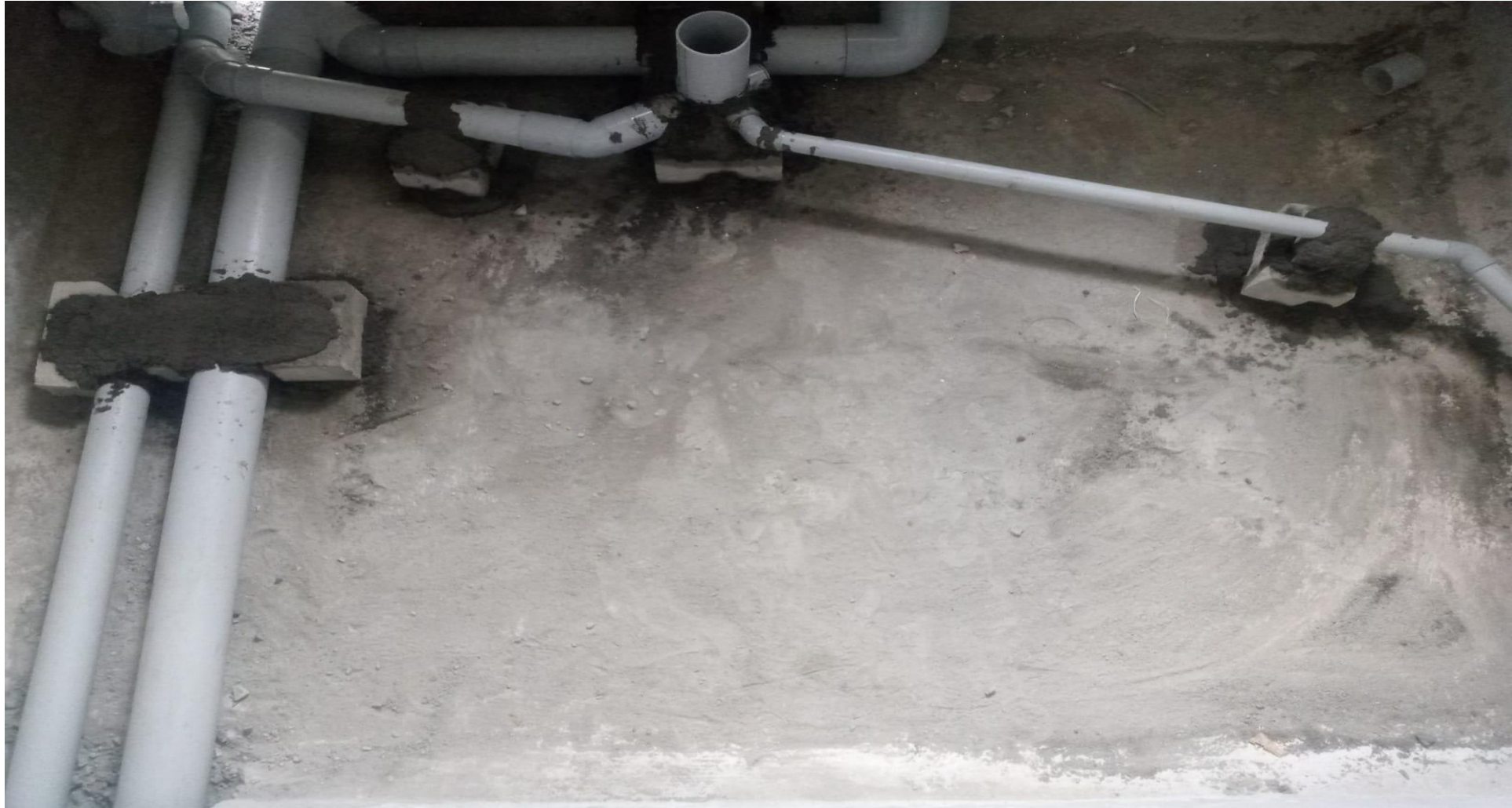
Villa No 11-SFToilet Soil and Waste Line Pipe Laying Work On Progress.
