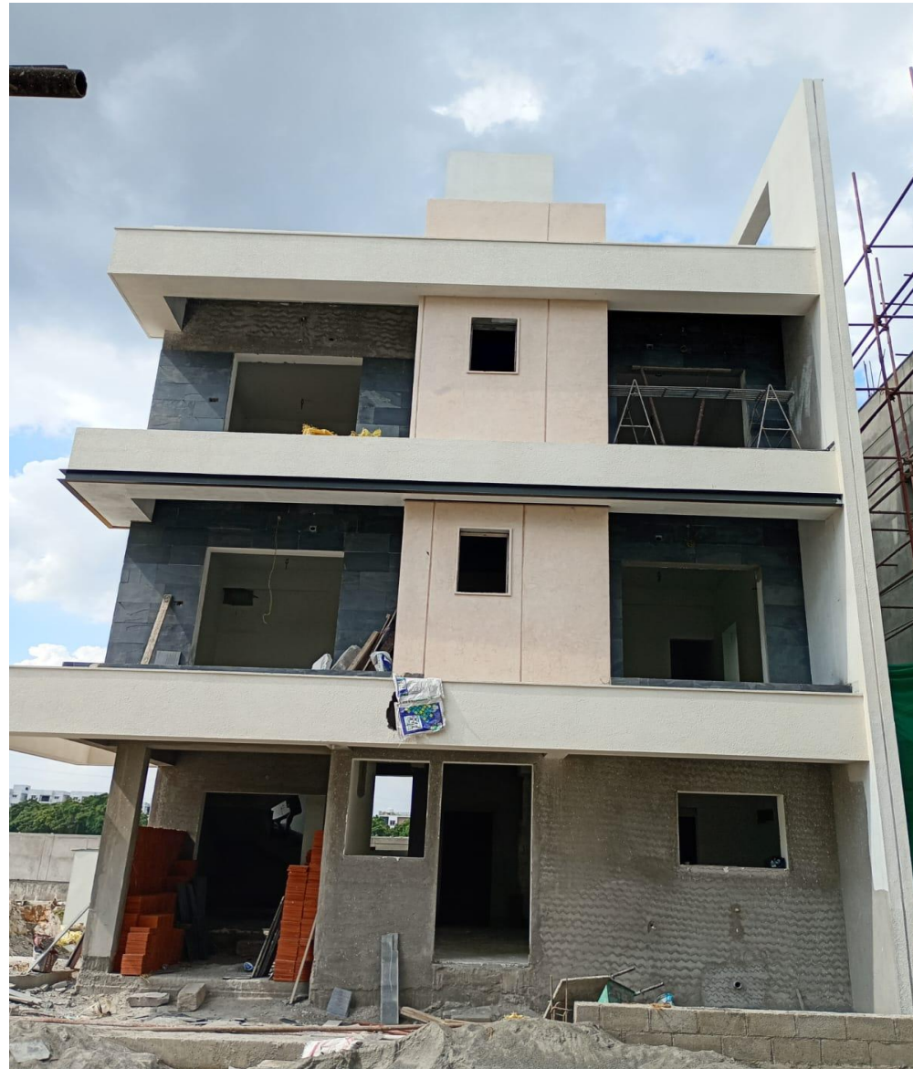
Villa No 12- Front Elevation Slate Tiles Laying Work In Progress
