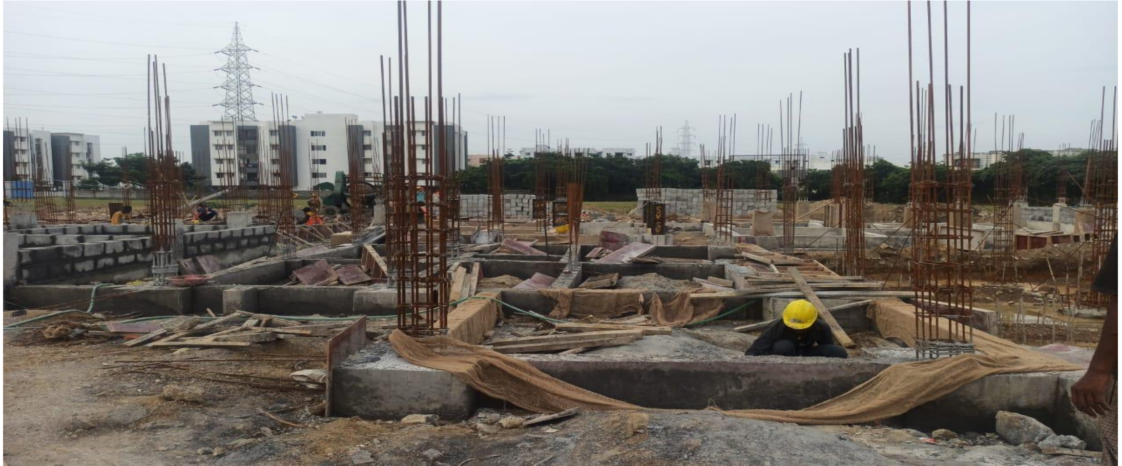
Phase 2 – villa no 69 Plinth Beam Concrete Completed
