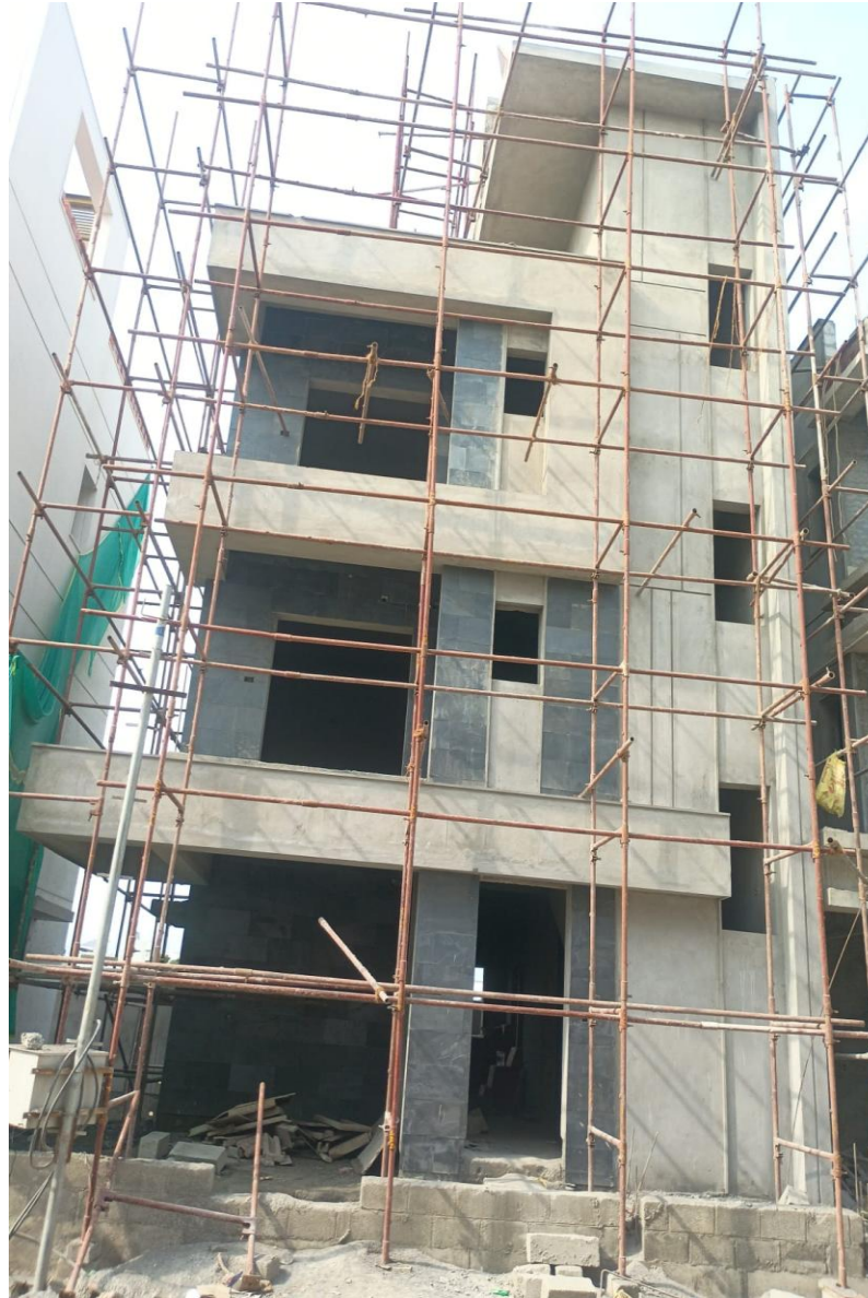
Villa No 13- Front Elevation View
