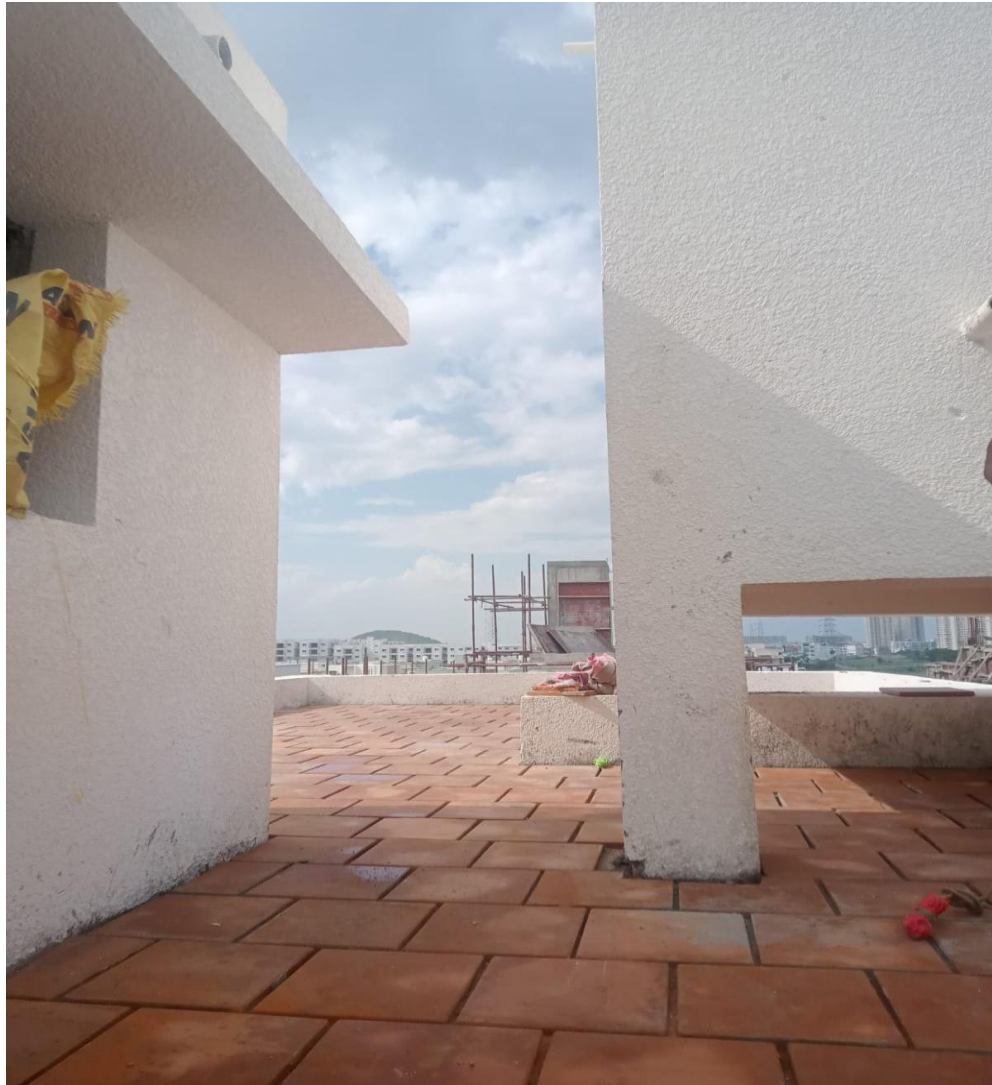
Villa No9 –Terrace Area Clay Tiles Laying Completed
