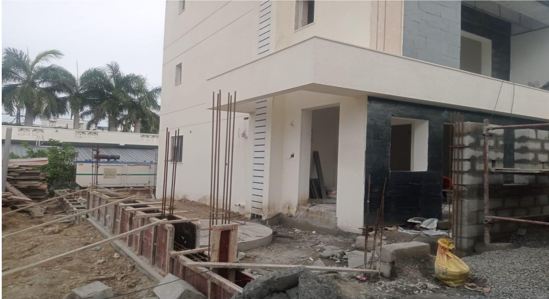
Villa No 3-Compound Wall Plinth Beam Shuttering Work In Progress
