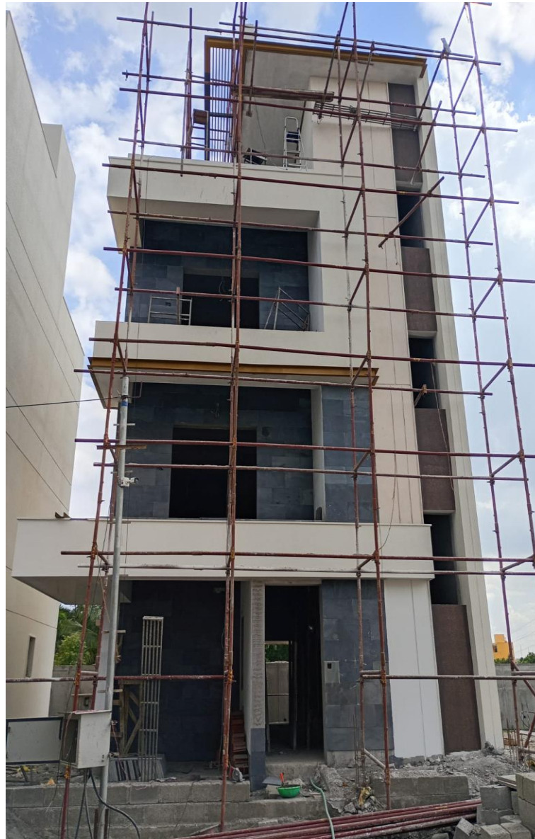
Villa No 11-Front elevation MS Pergola Fixing Work Completed
