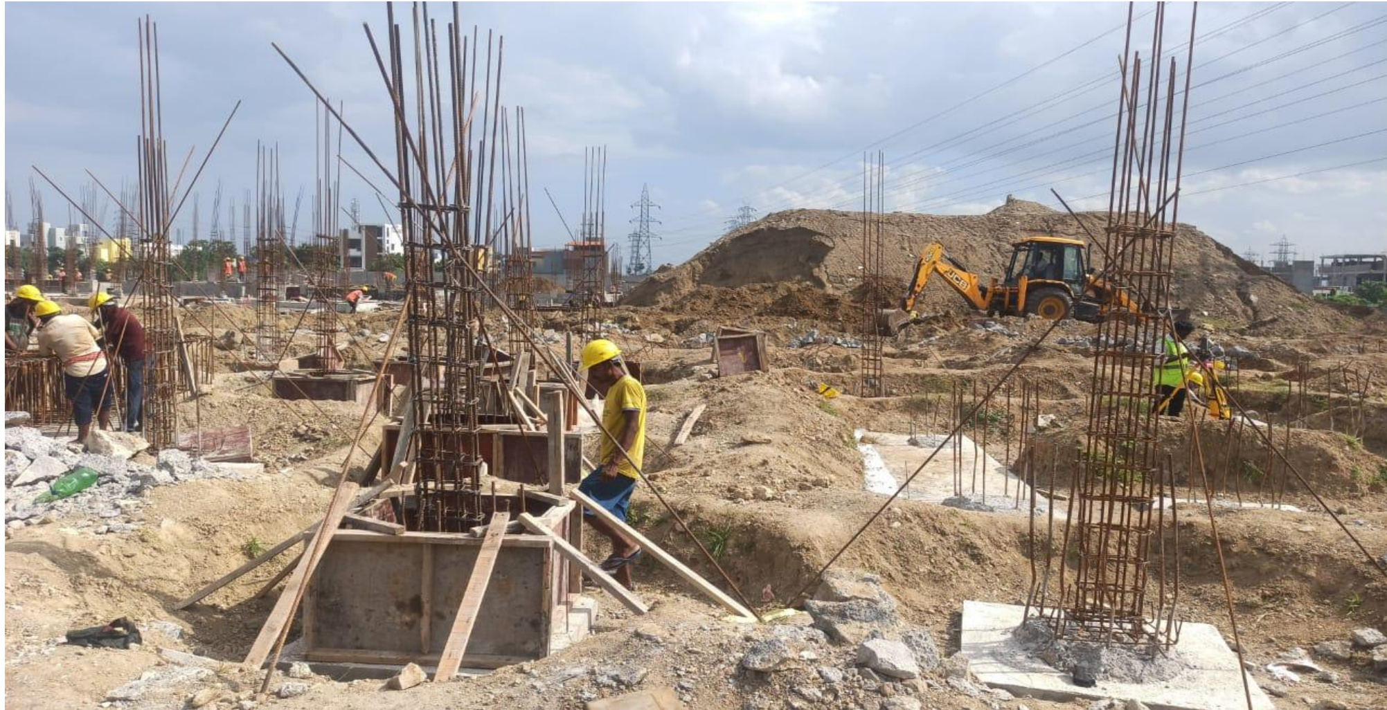
Phase 2 – villa no 80 Pile Cap Shuttering Work In Progress
