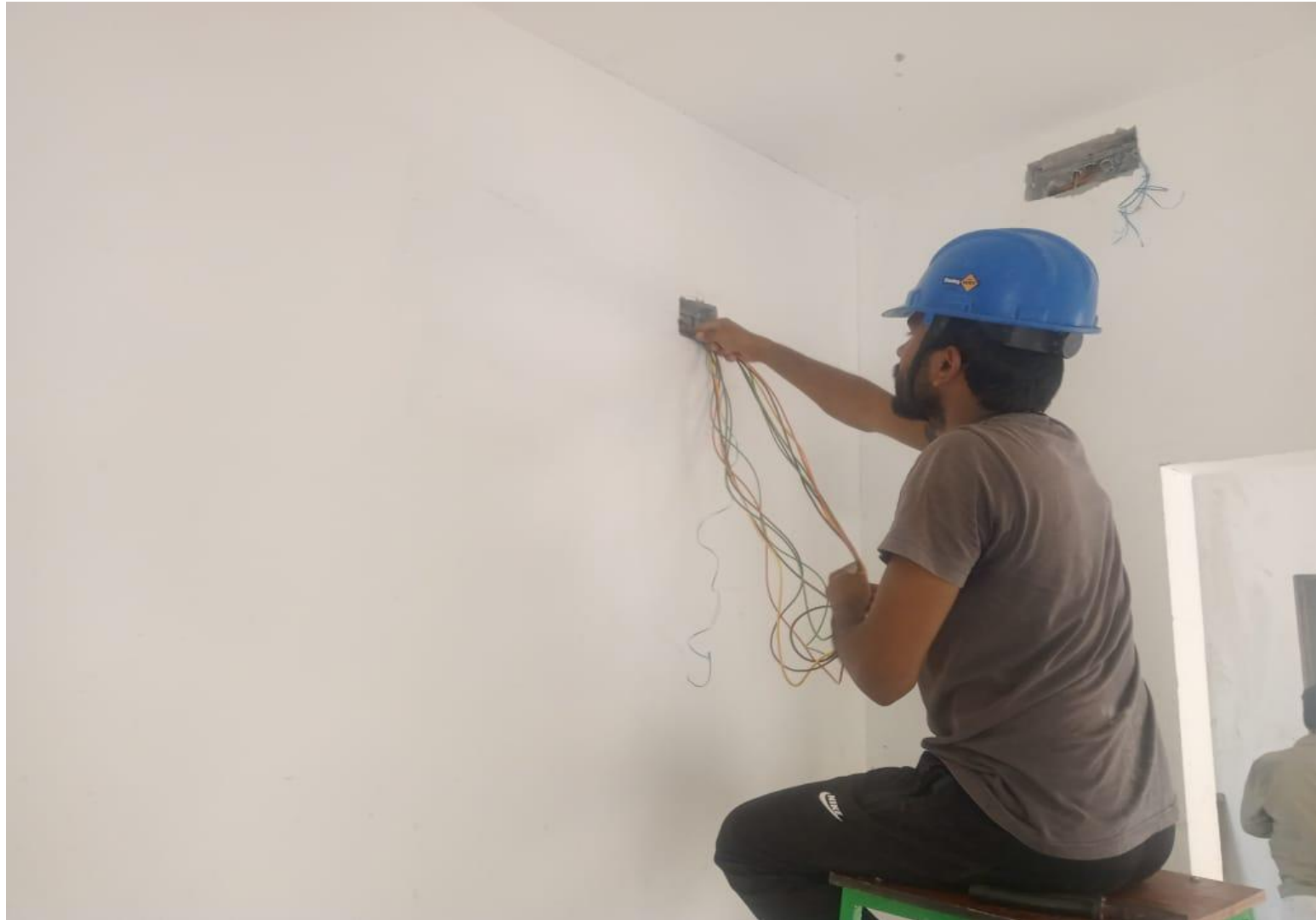
Villa No - 5 Wire Pulling Work Progress
