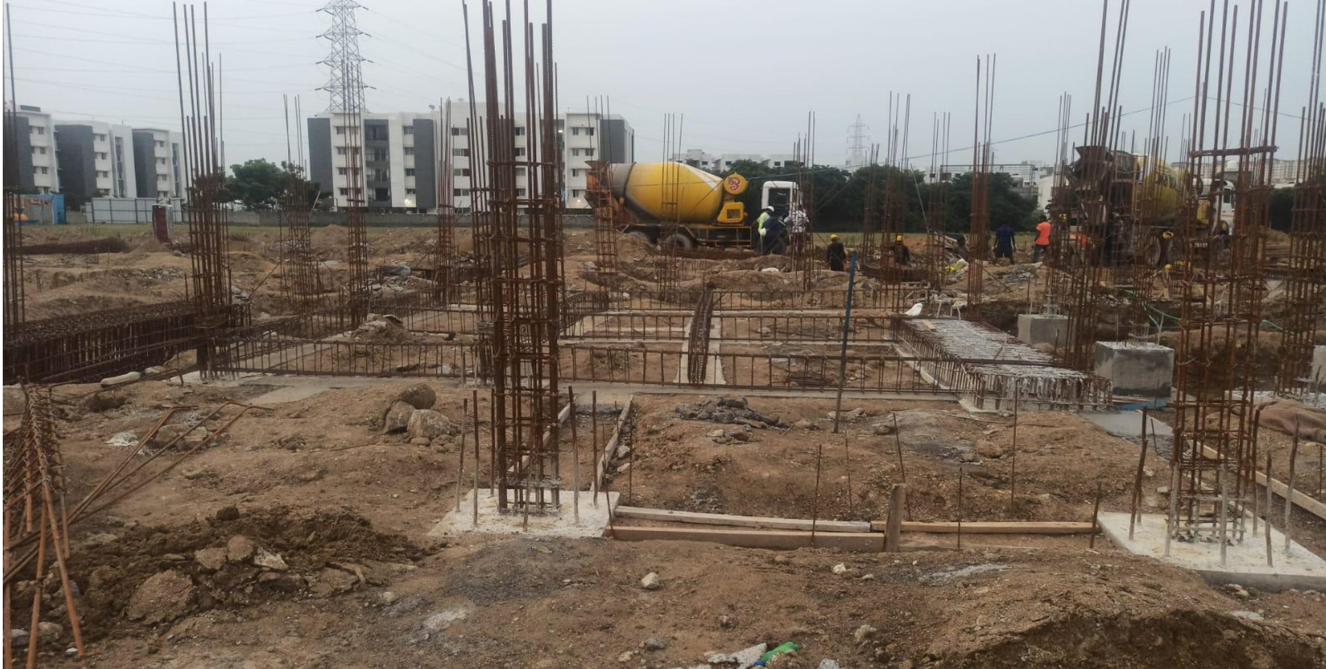
Phase 2 – villa no 68 Plinth Beam Reinforcement Work In Progress
