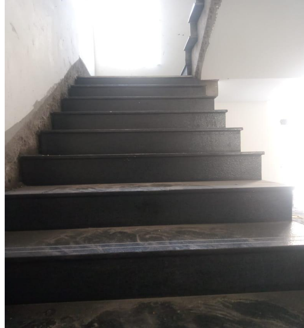
Villa No 7-Staircase Granite Laying Work Completed
