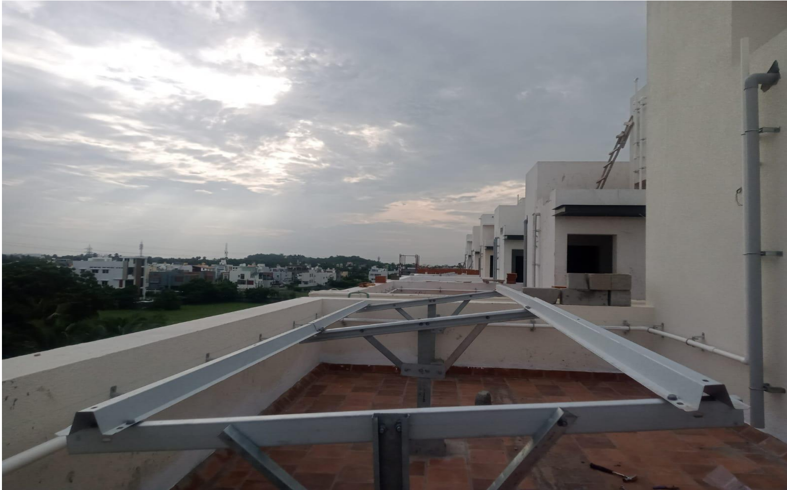
Villa No 6- Solar Panel Channel Fixing Work On Progress
