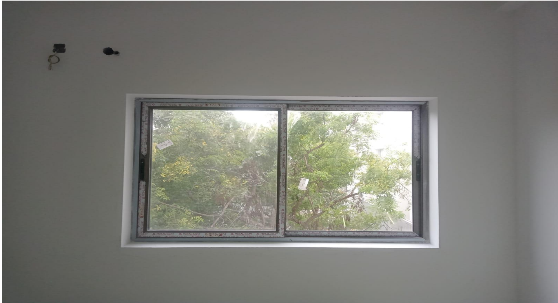
Villa No 4-Window Fixing Work Progress
