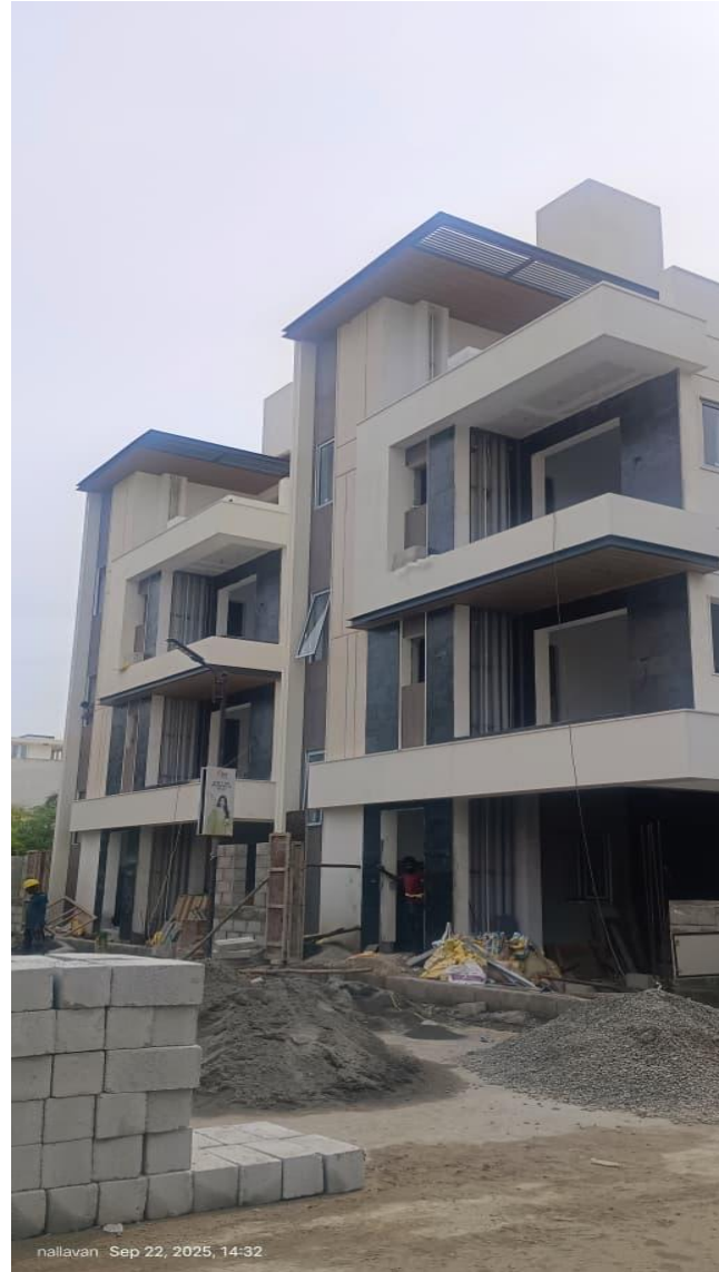
Villa No 4 & 5 Side Elevation view
