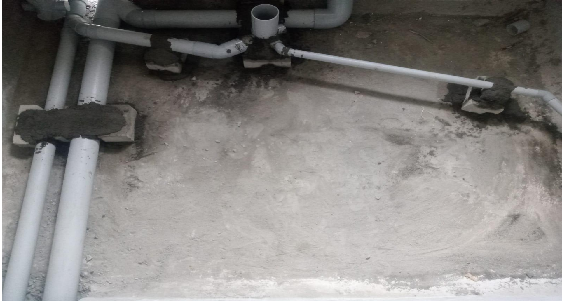
Villa No 13-SFToilet Soil and Waste Line Pipe Laying Work On Progress.
