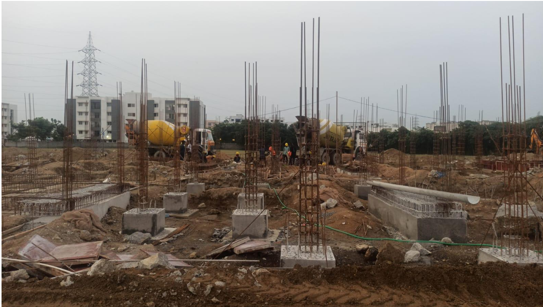
Phase 2 – villa no 69 Pile Cap Concrete Completed
