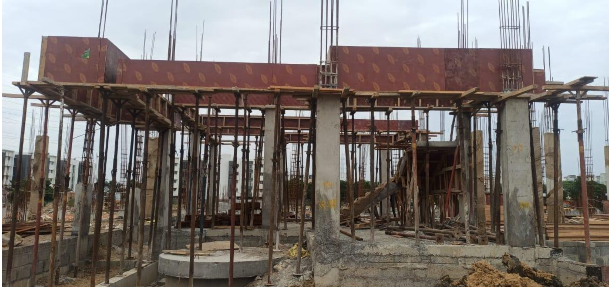
Phase 2 – villa no 49 GF Roof Slab Shuttering Work In Progress
