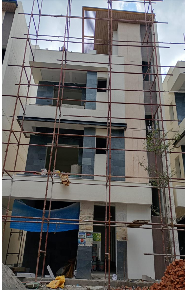
Villa No 7-Front elevation MS Pergola Fixing Work Completed
