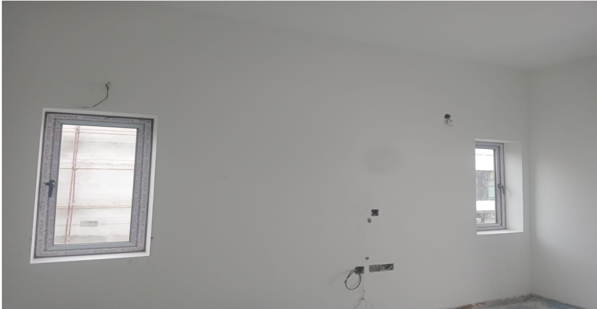
Villa No -5 Window Fixing Work Progress
