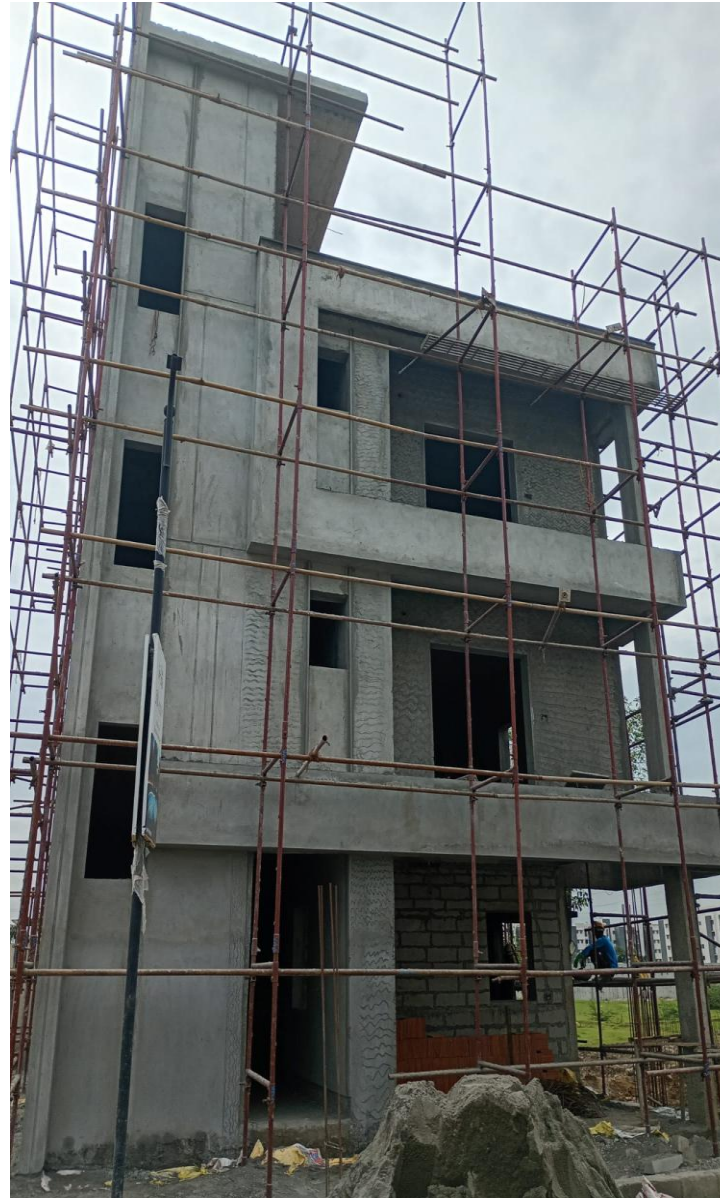
Villa No 17–East Side External Plastering Work Completed
