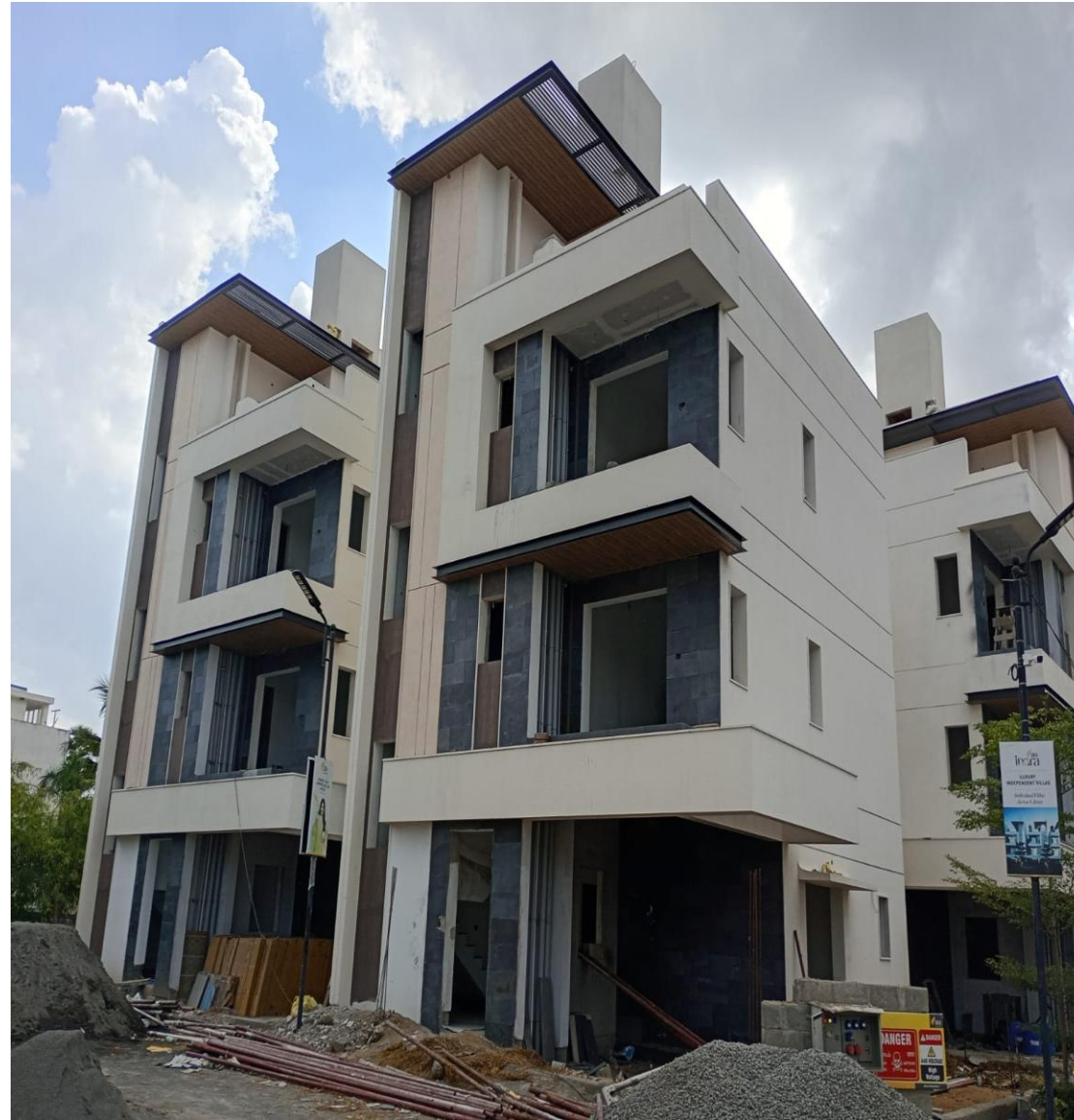
Villa No 4 & 5 Side Elevation view
