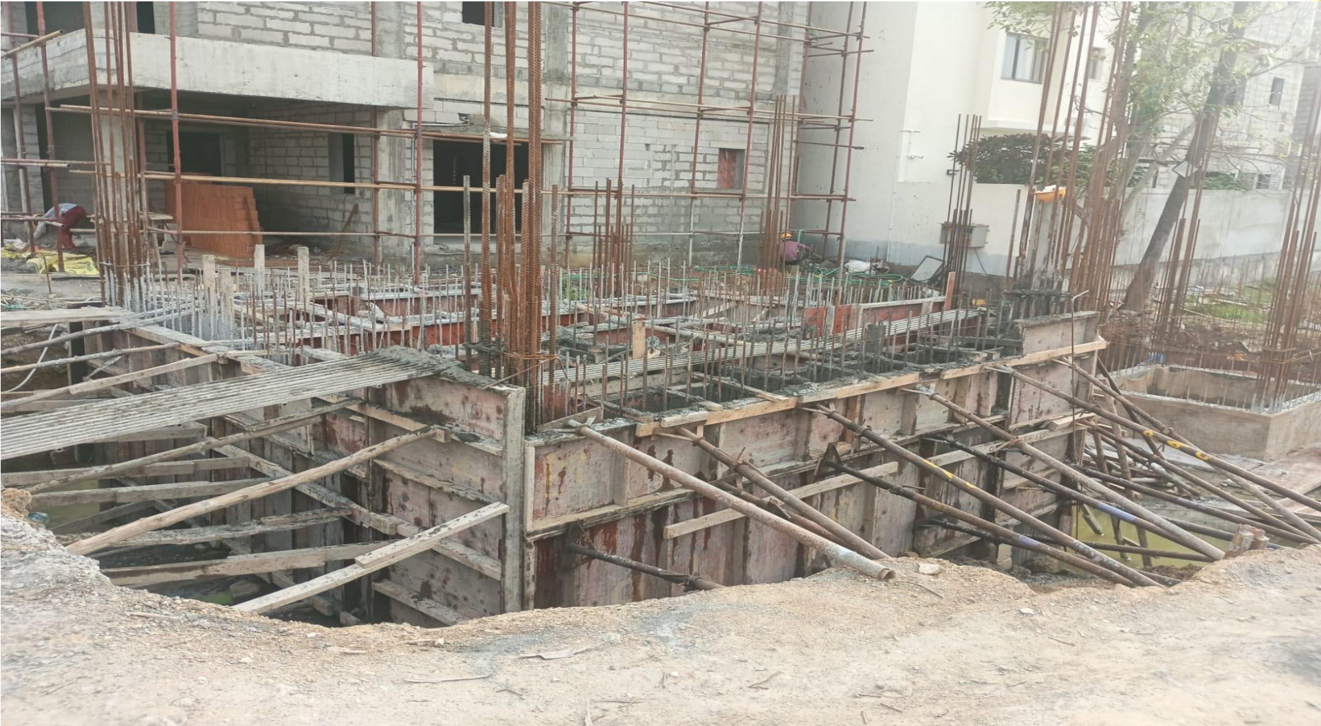
Villa No-18&19 STP RCC Wall Concrete Pouring Completed
