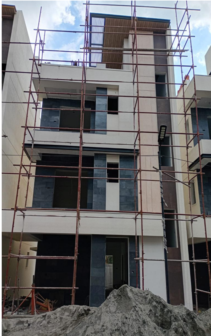
Villa No 8- Front elevation MS Pergola Fixing Work Completed
