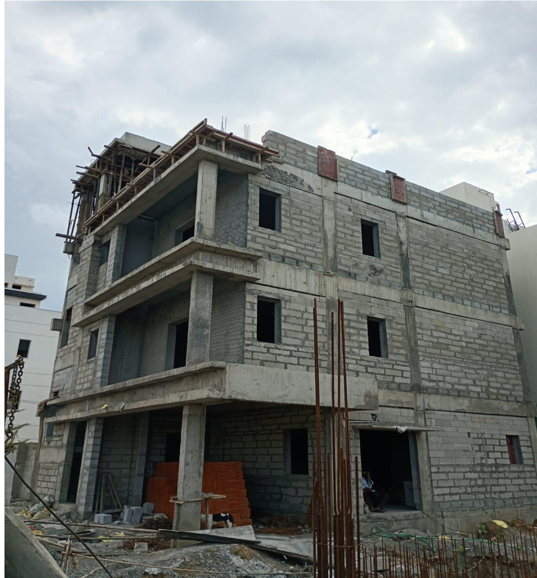
Villa No-17 Side Elevation View
