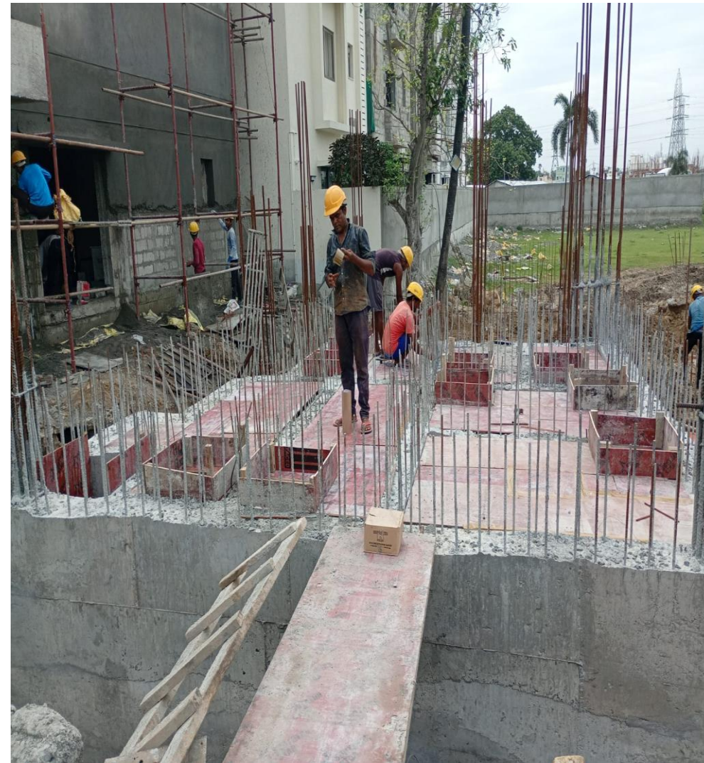
Villa No-18&19 STP RCC Wall Cover Salb Shuttering Work In Progress
