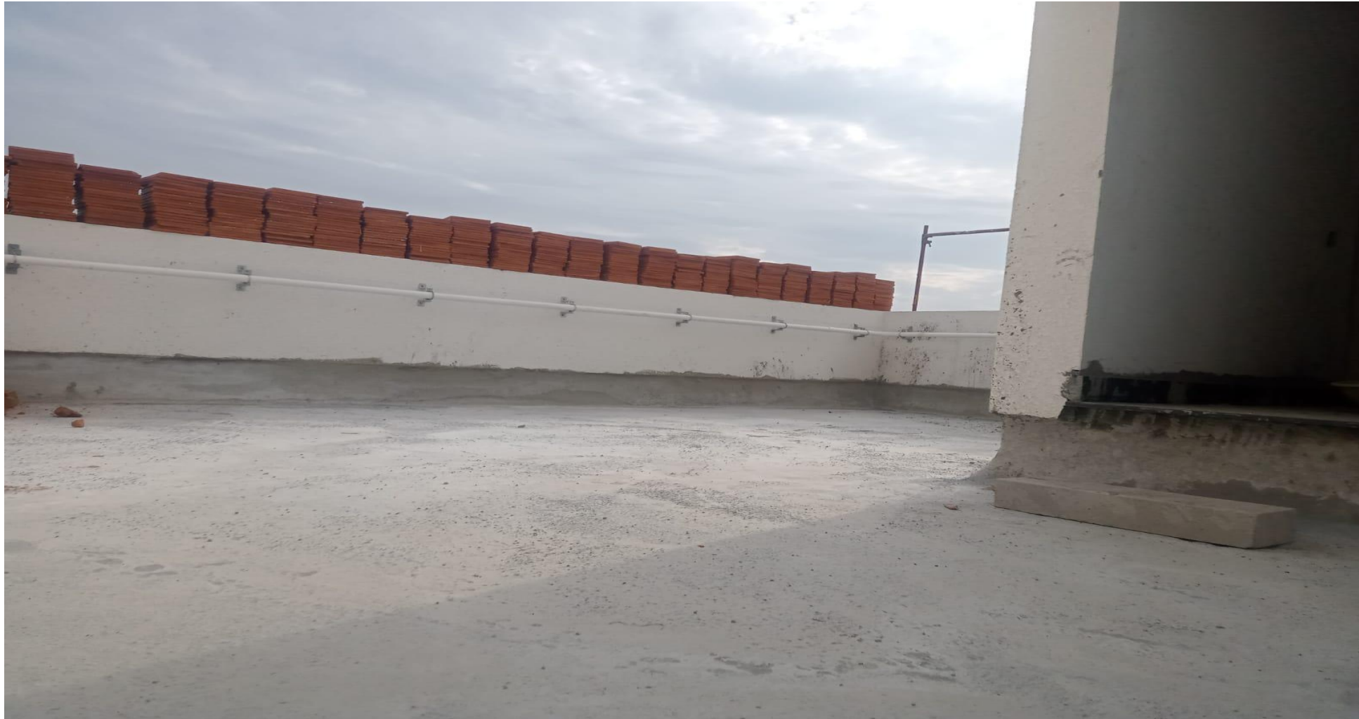
Villa No 10 –Terrace Area Waterproofing Protective Plastering Work Completed.
