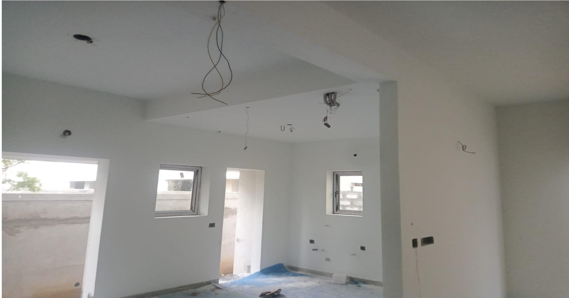
Villa No 4 - Second Coat Putty Scraping Completed
