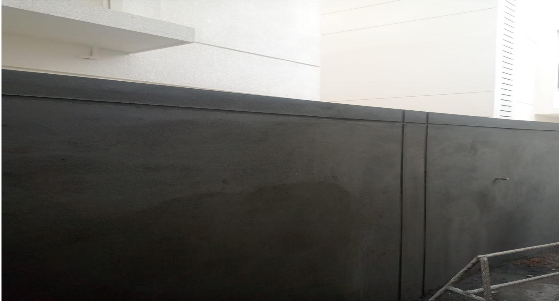
Villa No 6-Compound Wall Plastering Work In Progress
