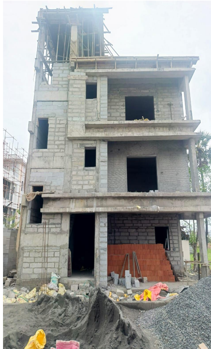
Villa No-17 Front Elevation Head Room Concrete Pouring Completed
