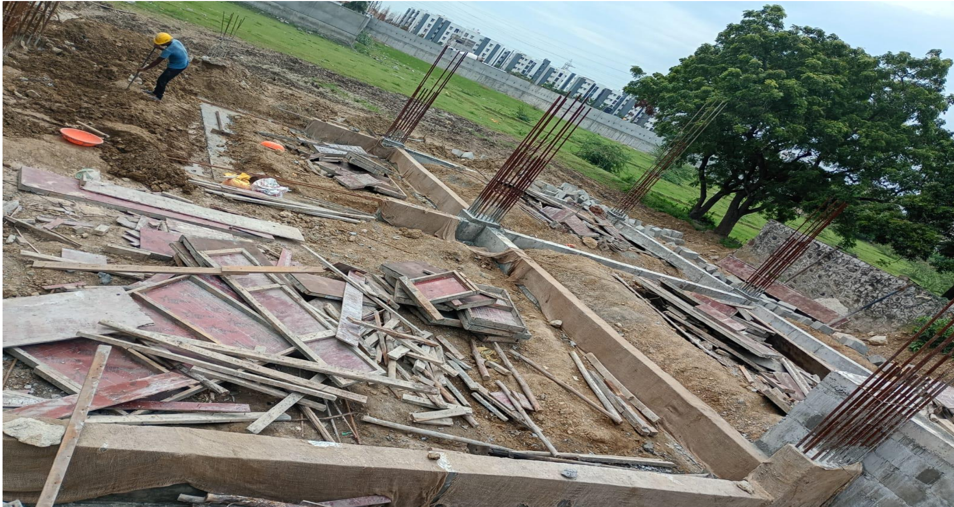
Villa No-18&19 Club House Plinth Beam Concrete Completed
