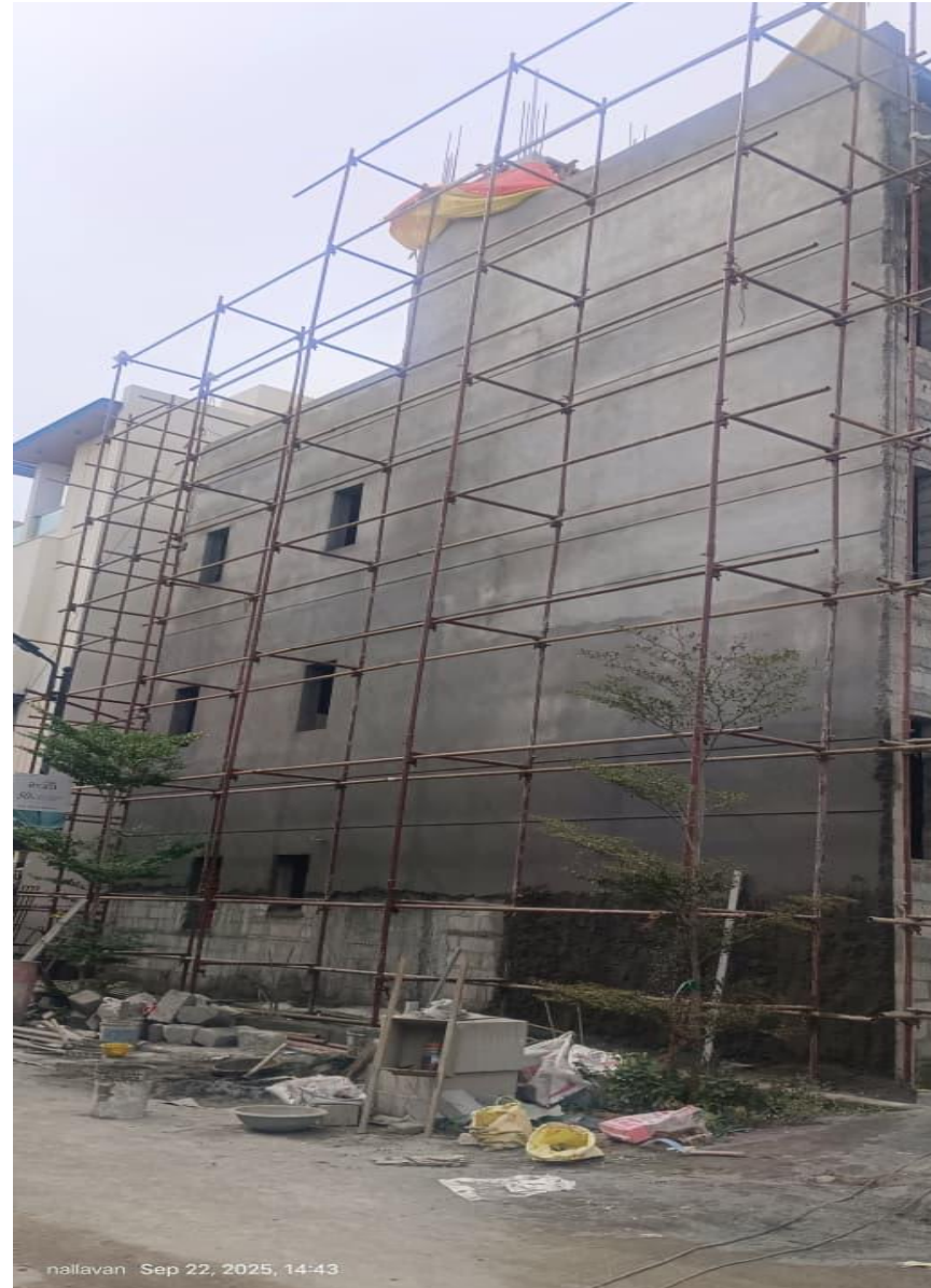
Villa No 17–South Side External Plastering Work In Progress
