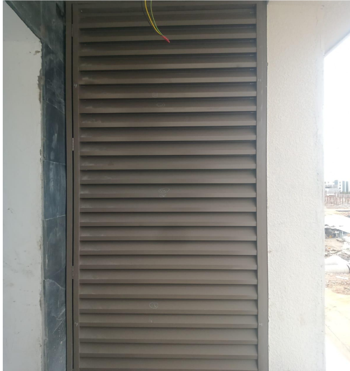
Villa No 9 –Aluminium Louvers Fixing Work On Progress
