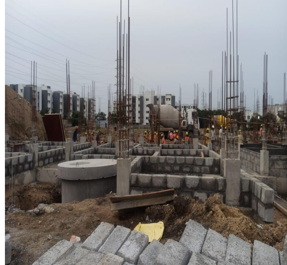
Phase 2 – villa no 47&48 Basement Block Work Completed
