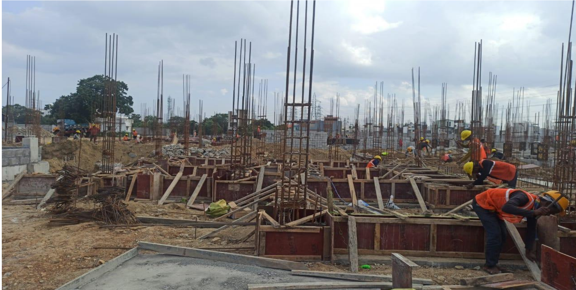
Phase 2 – villa no 74 Plinth Beam Shuttering Work In Progress
