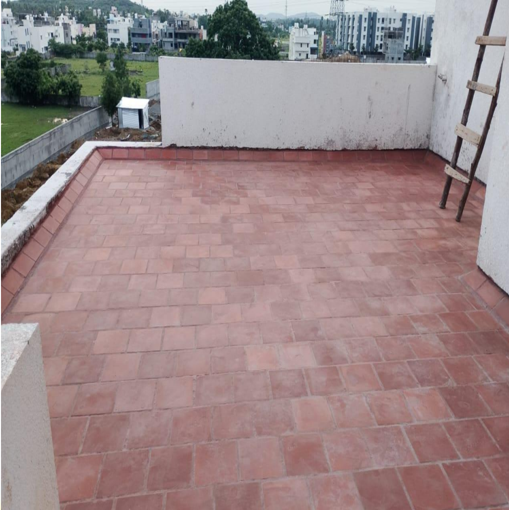
Villa No 12- Terrace Clay Tiles Laying Work Completed
