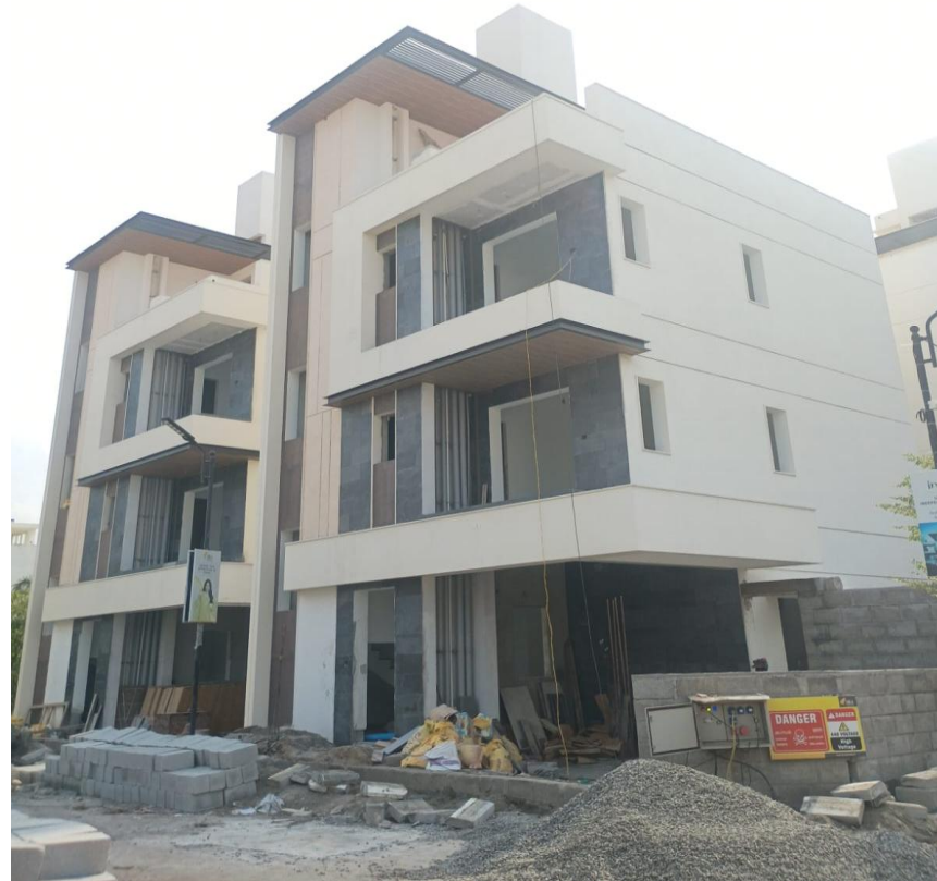
Villa No 4 & 5 Side Elevation view
