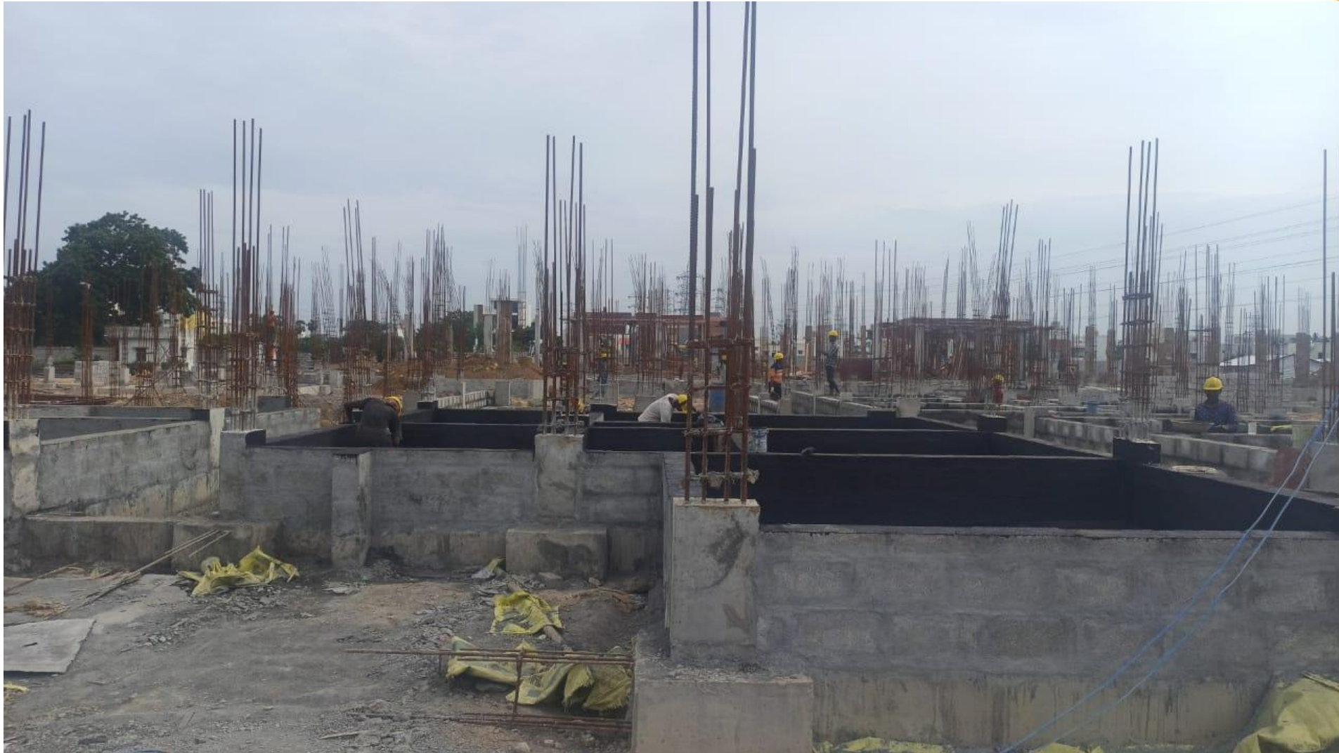
Phase 2 – villa no 75 Basement DPC Work In Progress
