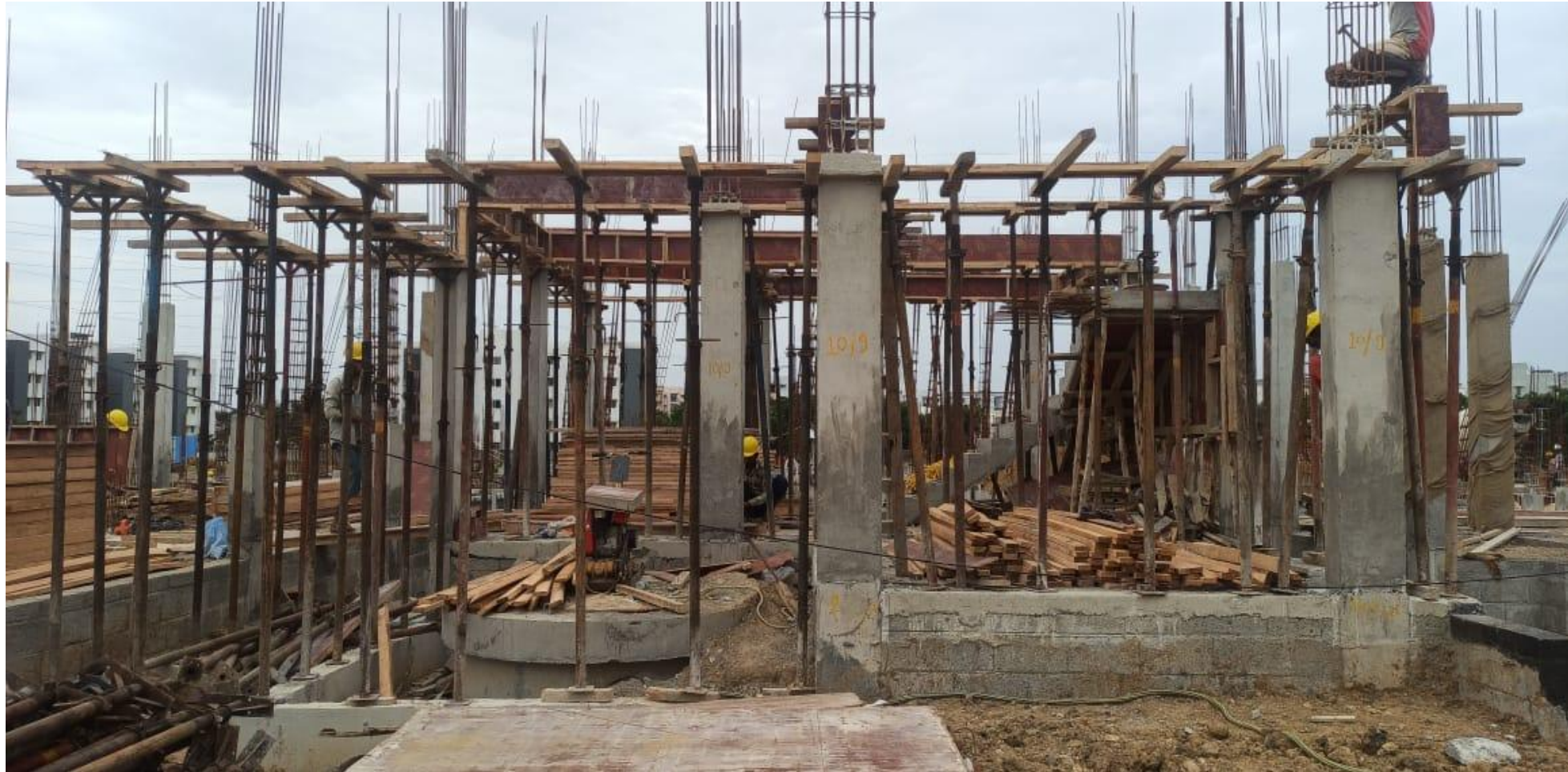
Phase 2 – villa no 51 GF Roof Slab Shuttering Work In Progress
