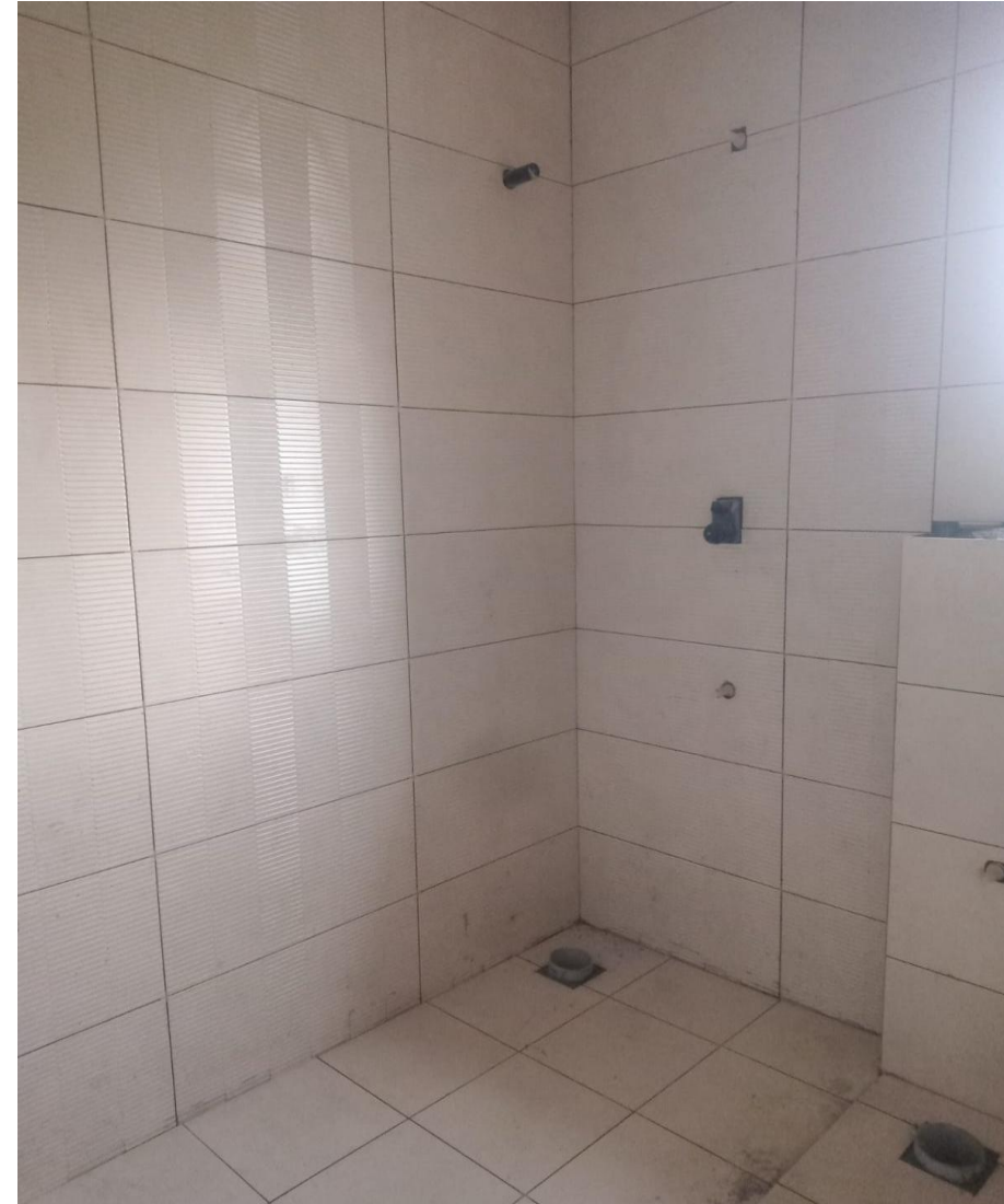
Villa No 8-FF&SF Toilets Tiles Laying Work In Progress
