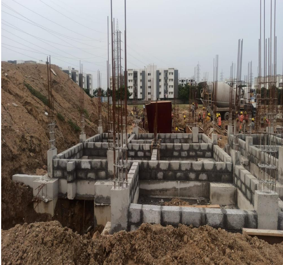
Phase 2 – villa no 47&48 Basement Block Work Completed
