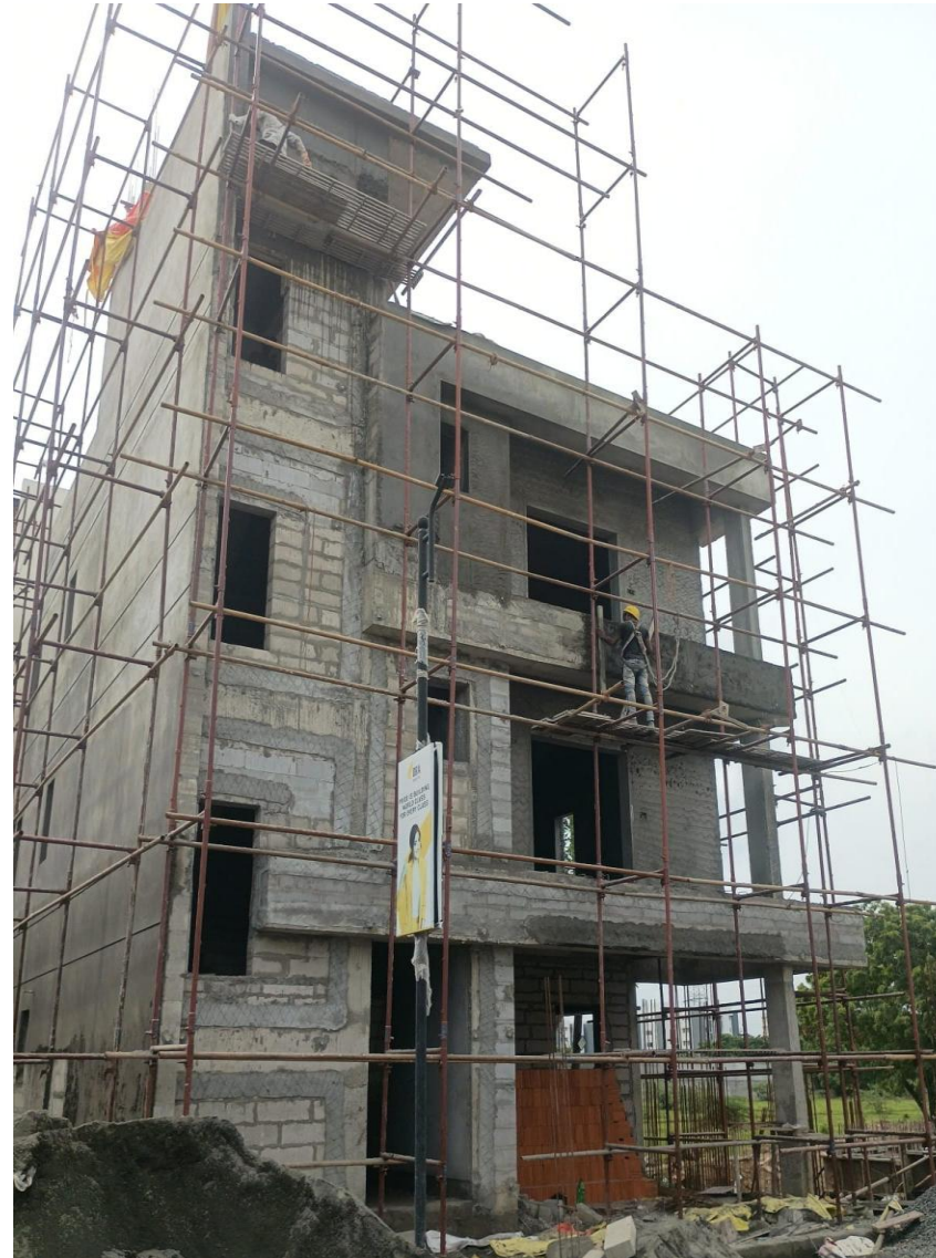
Villa No 17 –East Side External Plastering Work In Progress
