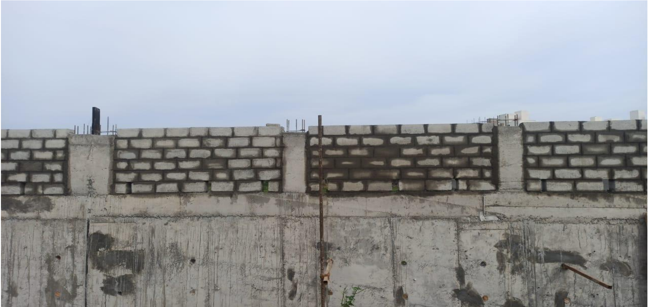
Phase 2 Compound Wall Block Work On Progress
