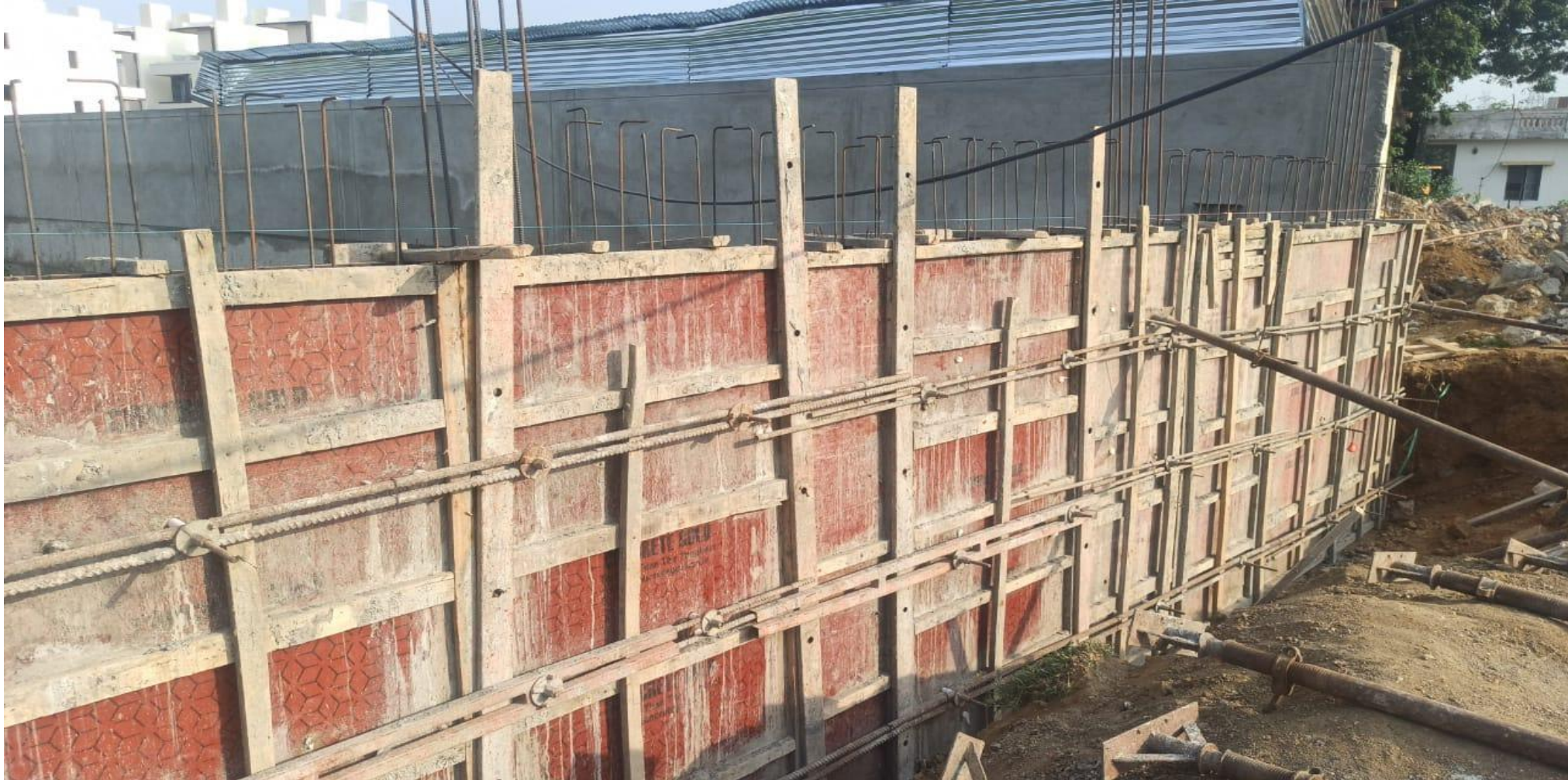
Phase 2 Compound Wall Shuttering Working On Progress
