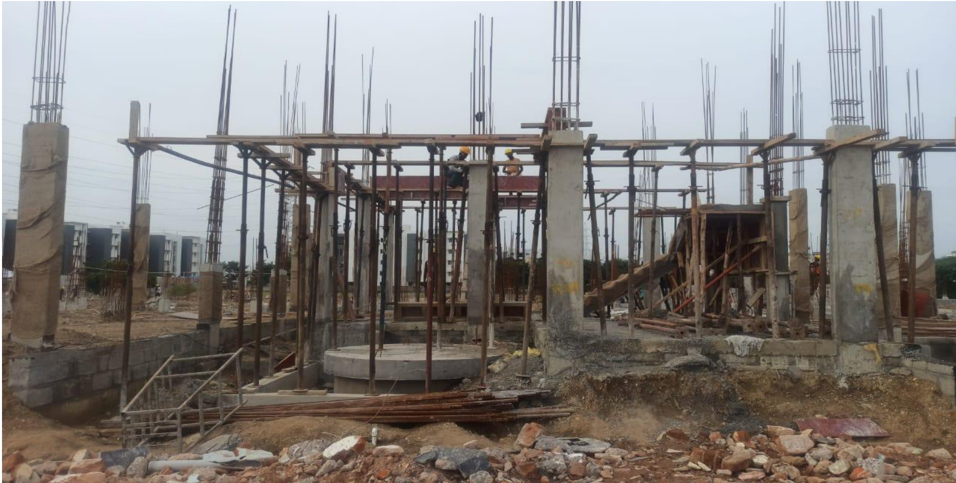
Phase 2 – villa no 49 GF Roof Slab Shuttering Work In Progress
