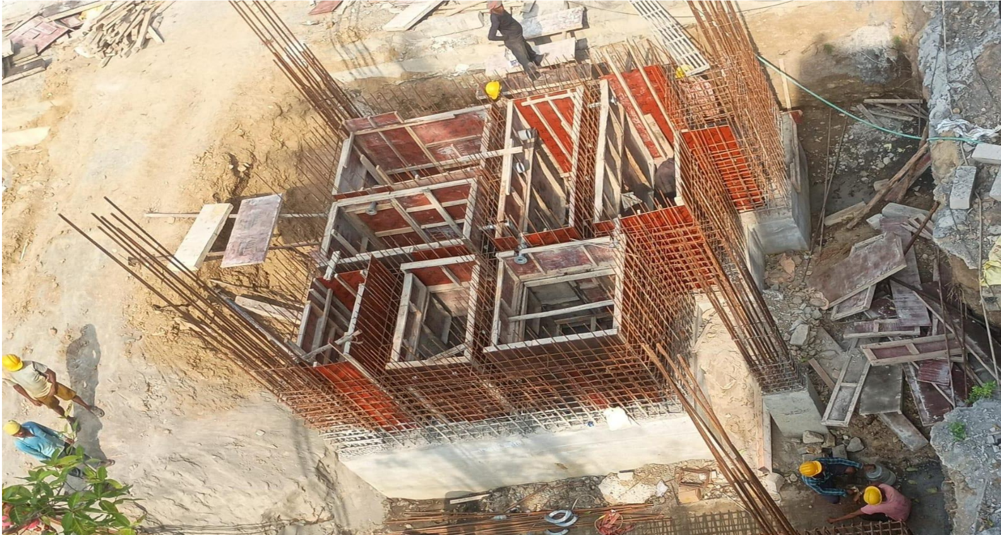
Villa No-18&19 STP RCC Wall Shuttering Working On Progress
