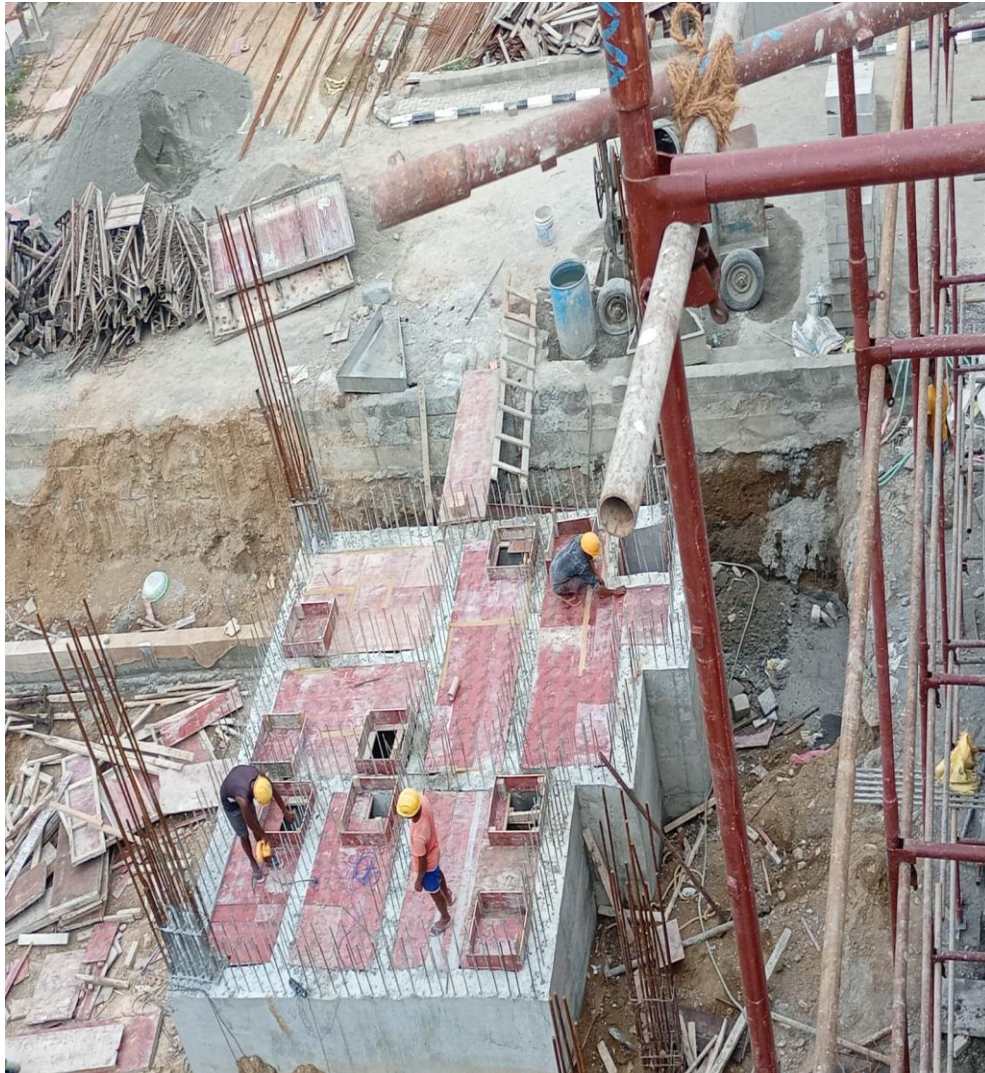
Villa No-18&19 STP RCC Wall Cover Salb Shuttering Work In Progress
