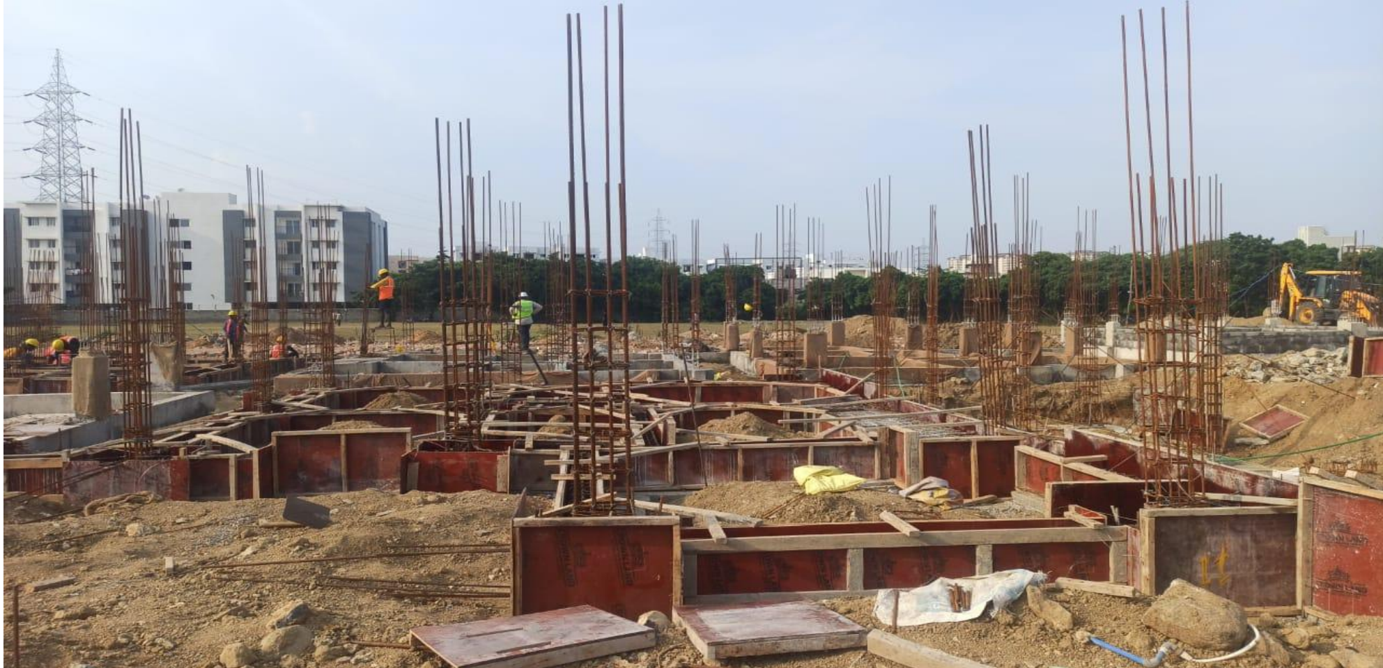
Phase 2 – villa no 69 Plinth Beam Shuttering Work In Progress
