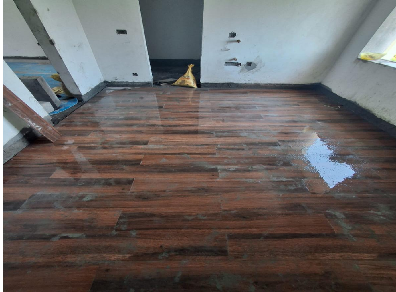
Villa No 9 –FF Bed Room Tiles Laying Work Completed
