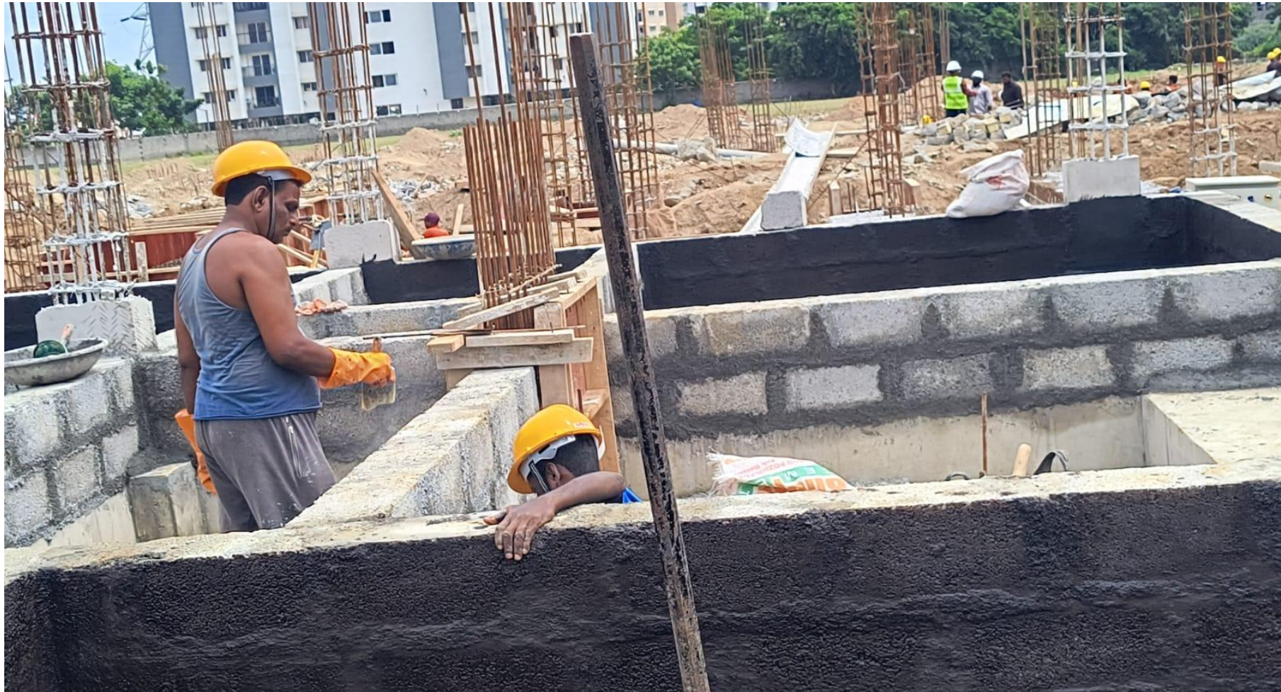
Phase 2 – villa no 50 Basement DPC Work In Progress
