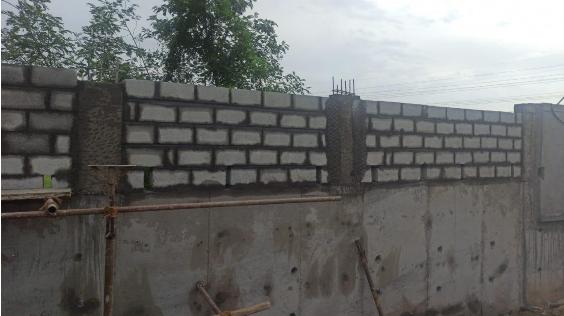
Phase 2 Compound Wall Block Work On Progress
