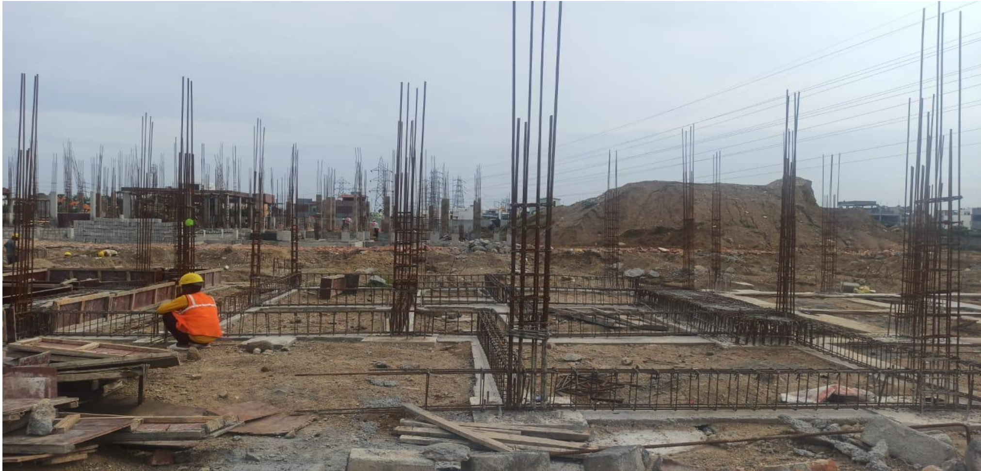
Phase 2 – villa no 79 Plinth Beam Reinforcement Work In Progress
