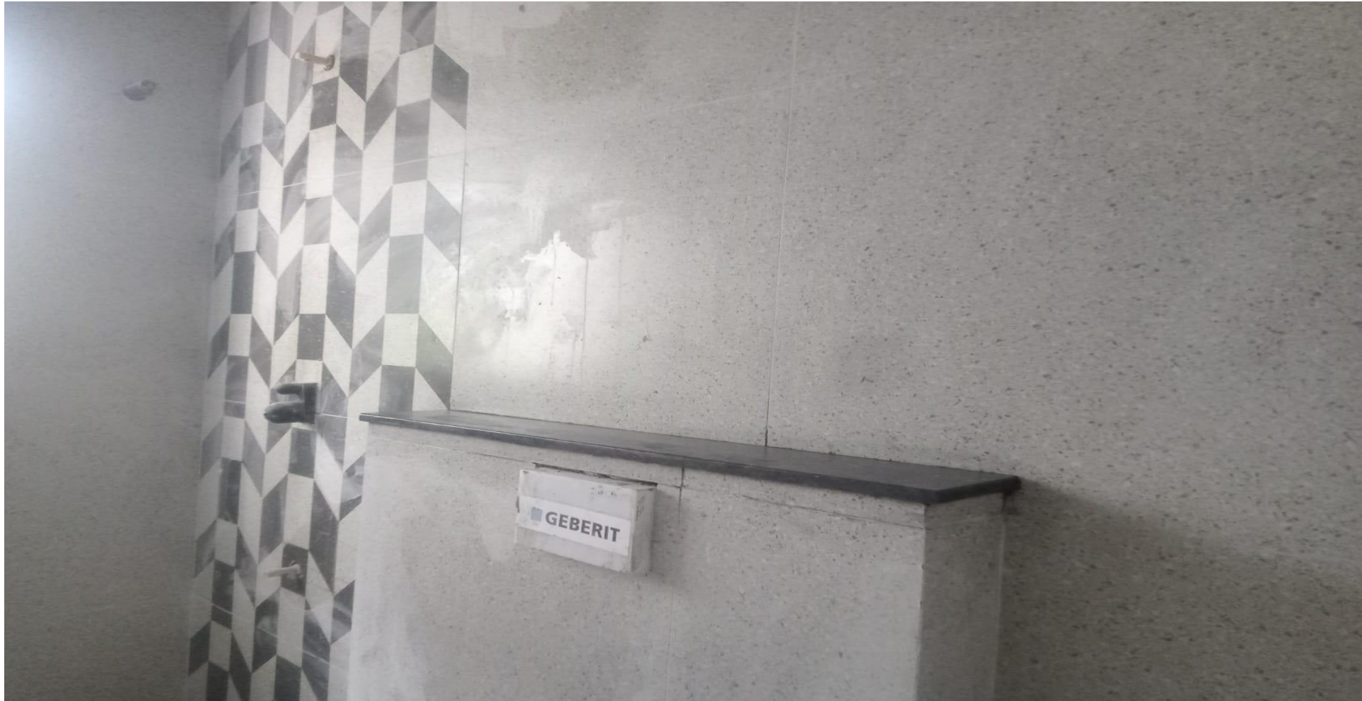
Villa No 3- Toilet Ledge Wall Threshold Granite Fixing Completed
