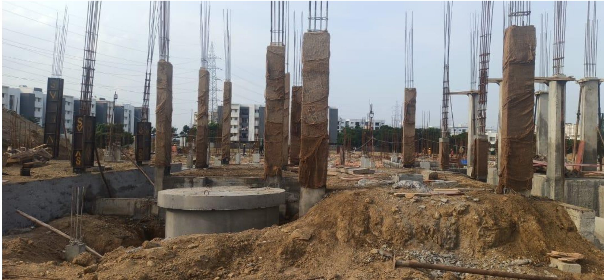
Phase 2 – villa no 48 GF Column Concrete Pouring Completed
