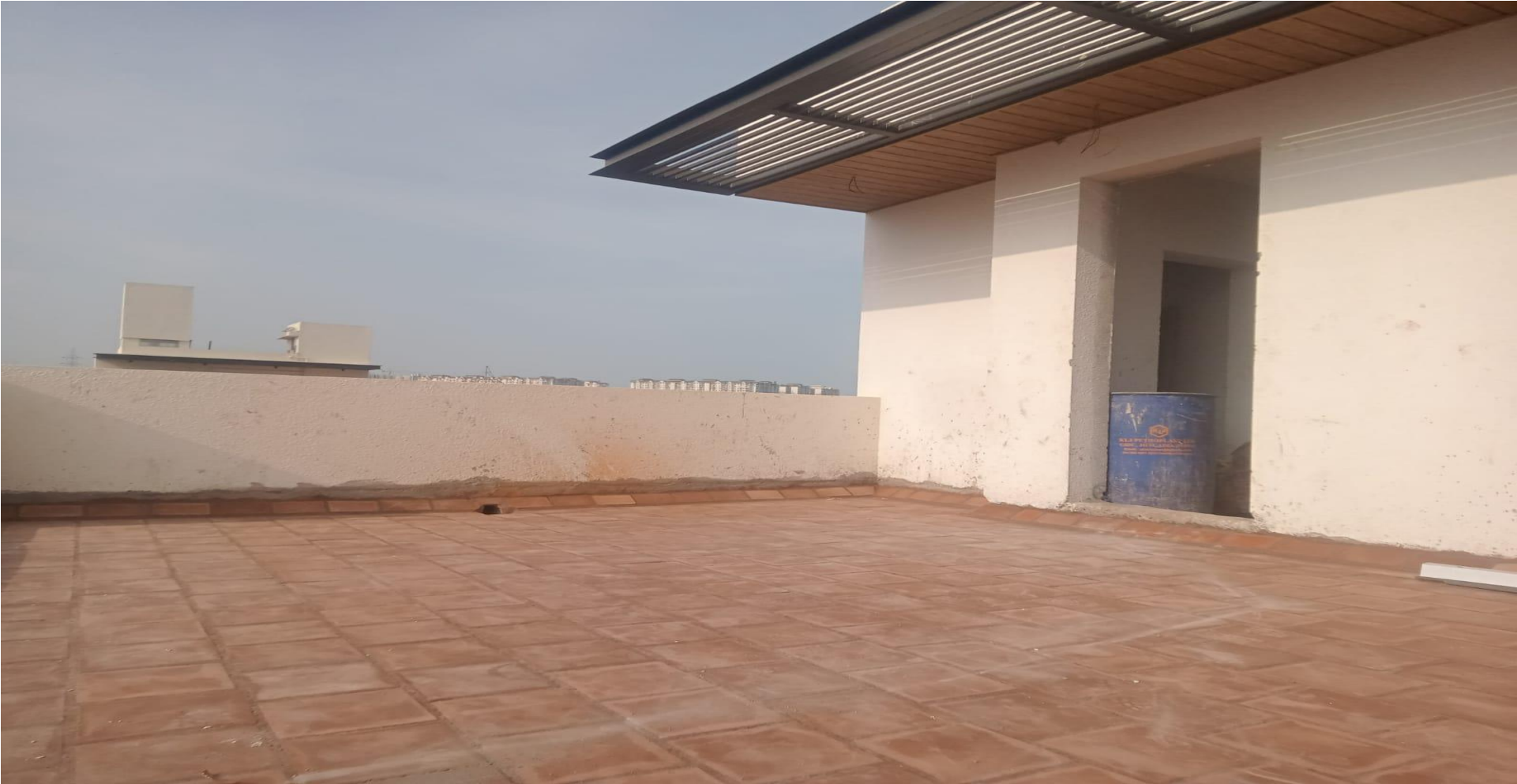
Villa No 3 Terrace Area Clay Tiles Laying Completed
