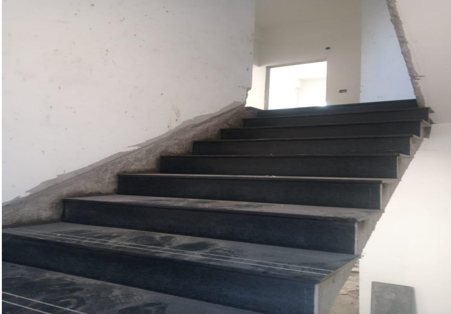
Villa No 10 –Staircase Granite Laying Completed
