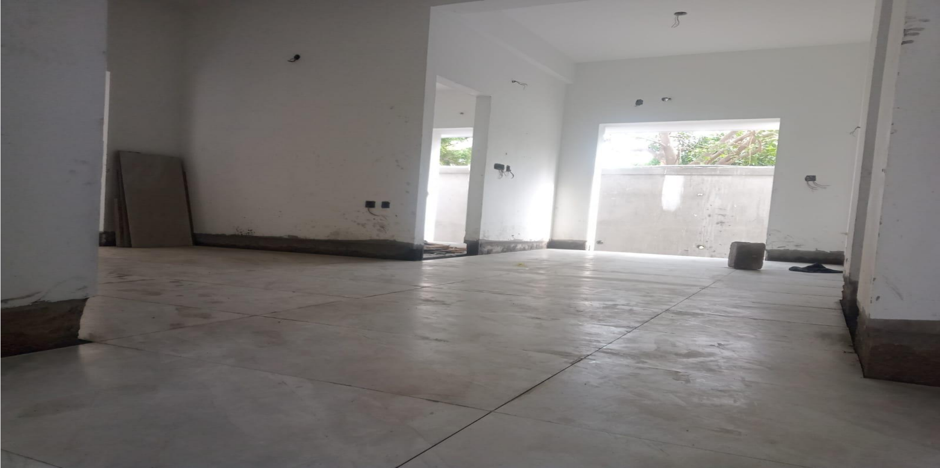
Villa No 7-GF Flooring Tile Laying Work Completed
