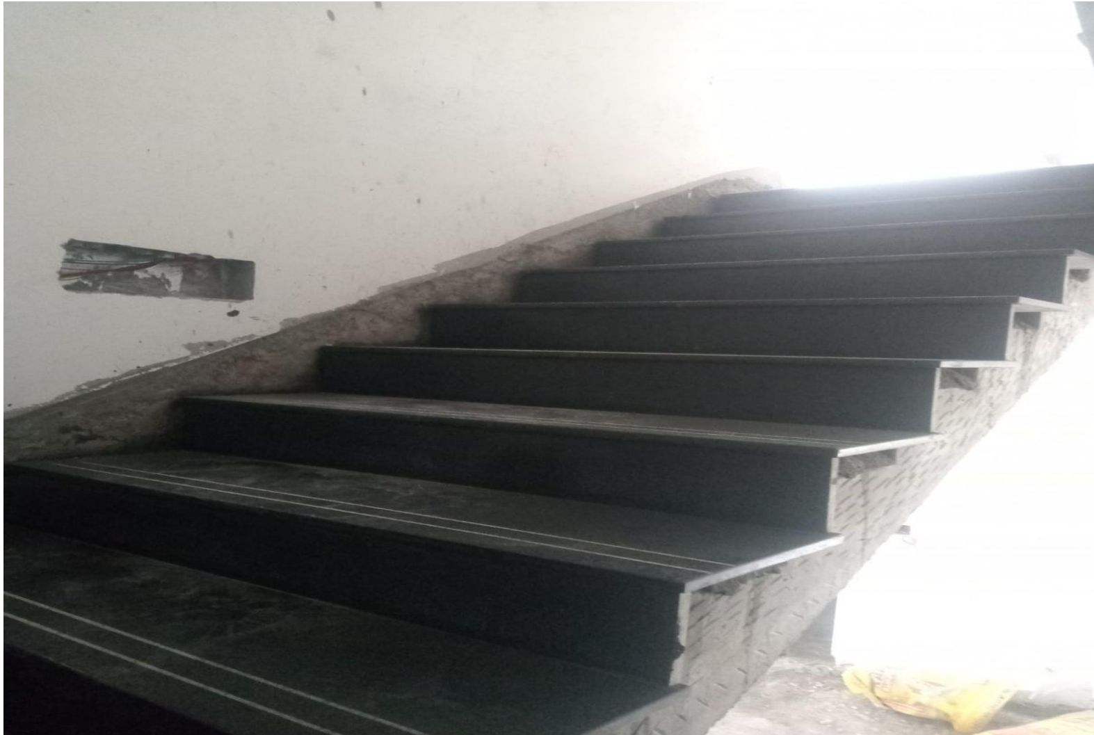
Villa No 3 Staircase Granite Laying Completed
