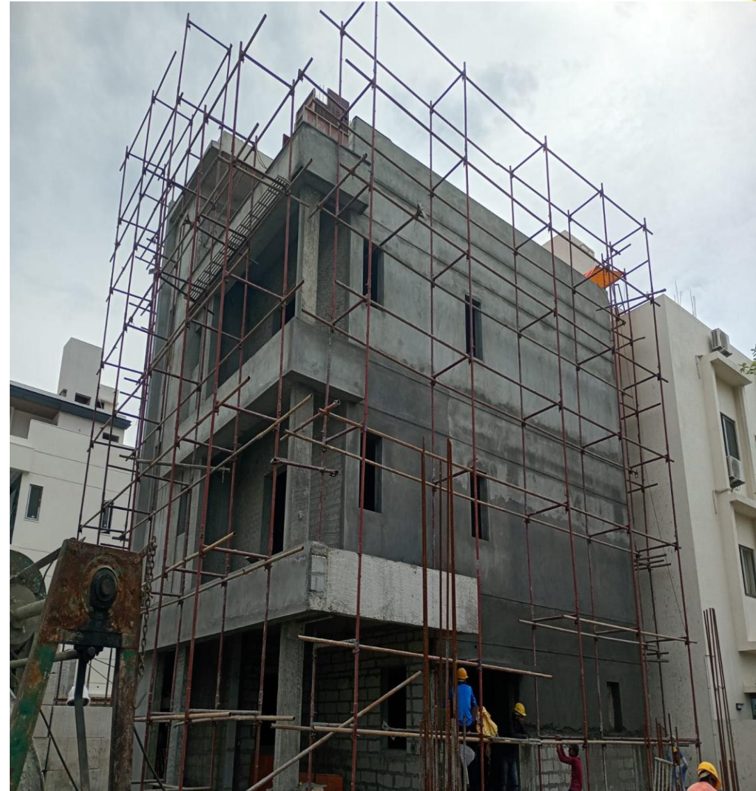
Villa No 17–South & North Side External Plastering Work In Progress
