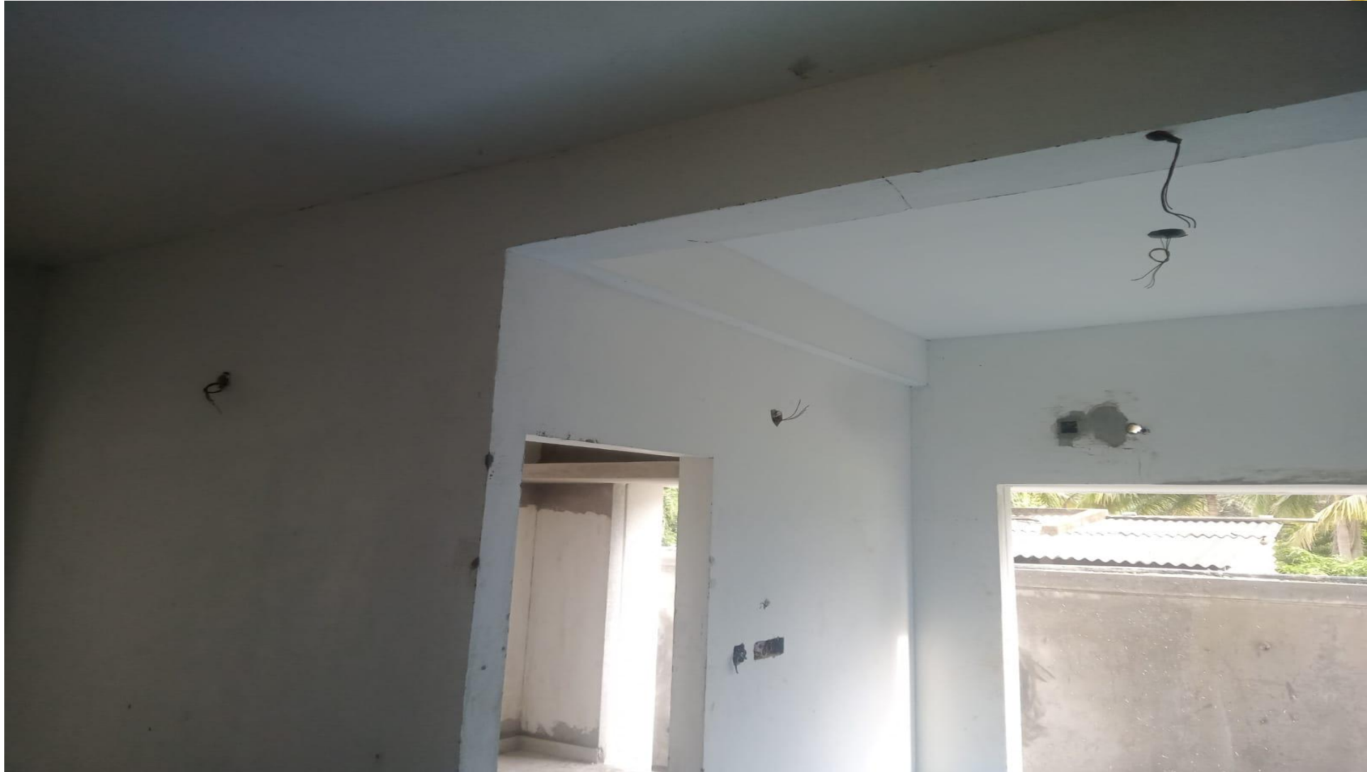
Villa No 9 – Electrical Wire Pulling Work On Progress
