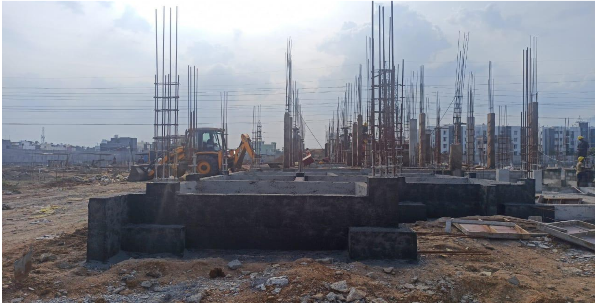
Phase 2 – villa no 53 Basement DPC Work Completed
