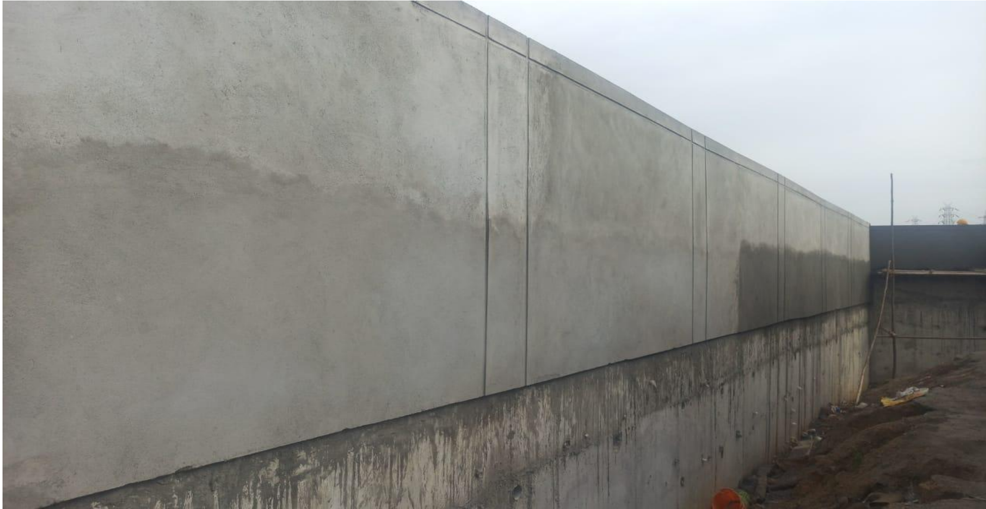
Phase 2 Compound Wall Plastering Work On Progress
