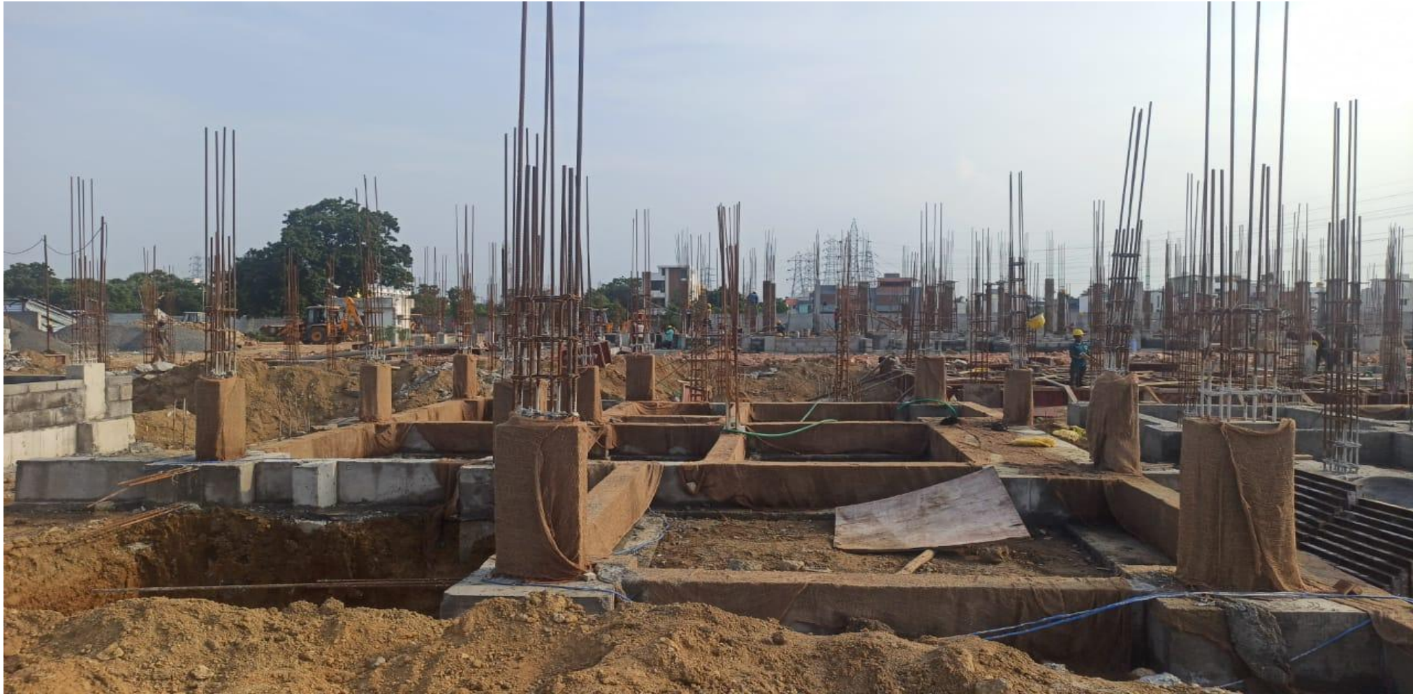
Phase 2 – villa no 74 Pedestal Column Concrete Completed
