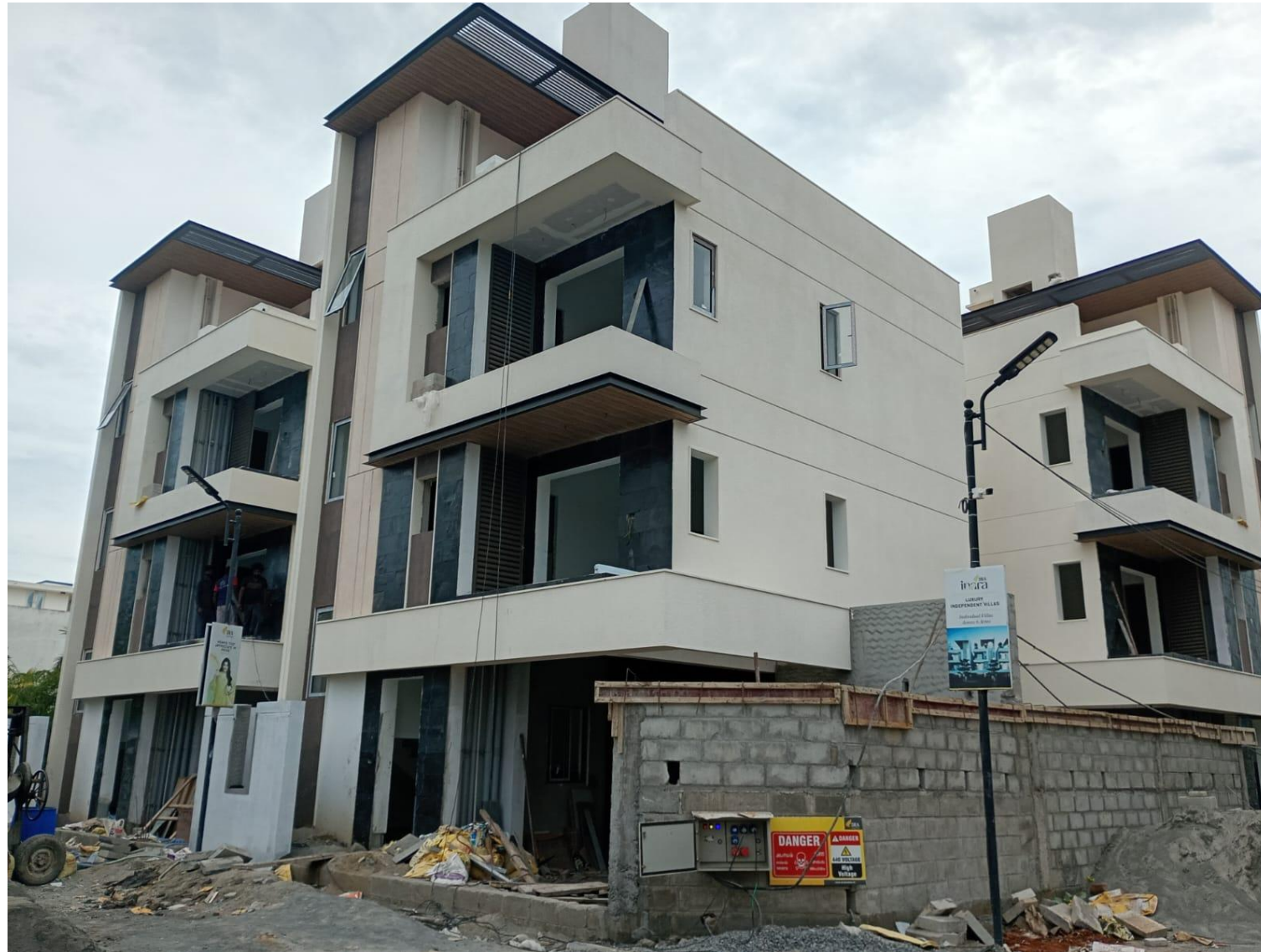
Villa No 4 &5&6 Side Elevation view
