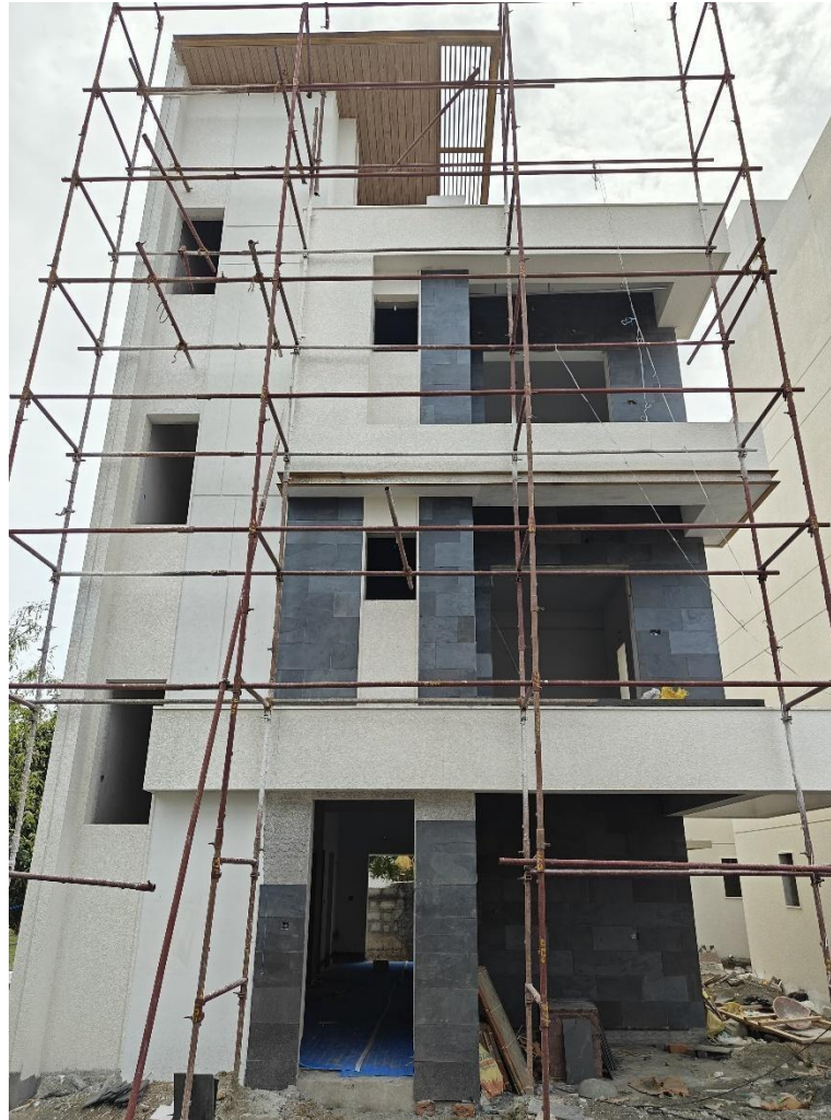
Villa No 4 – Front Elevation Slate tile laying work Completed
