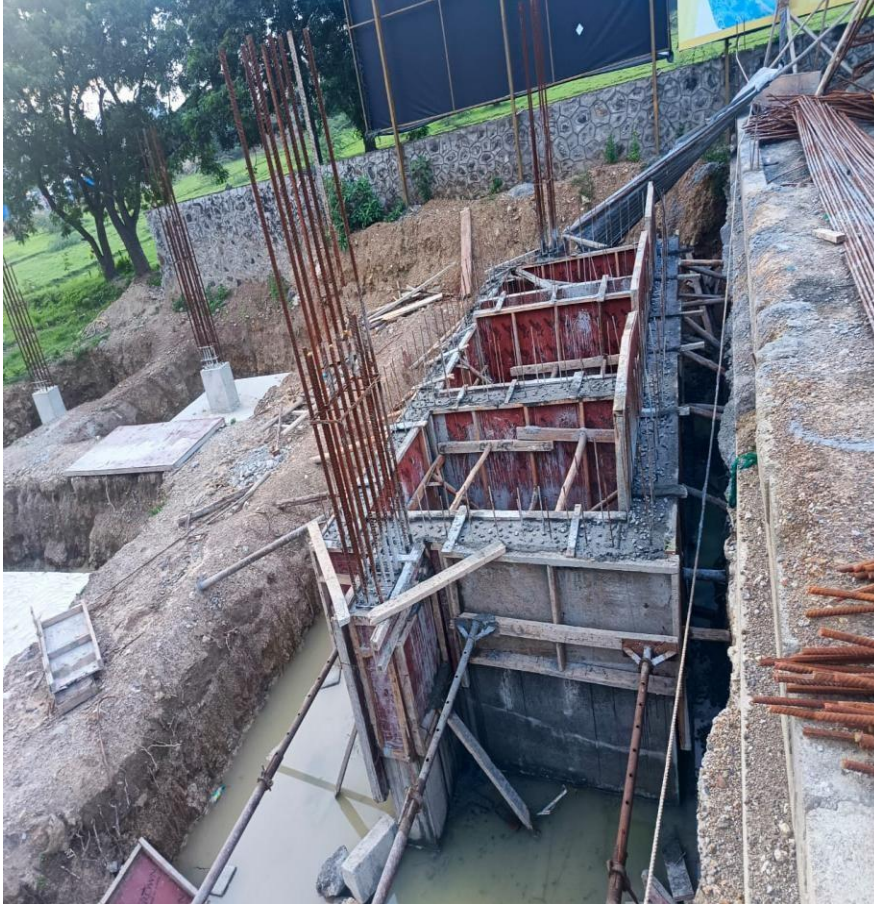
Villa No 18–UG Sump Concrete work completed
