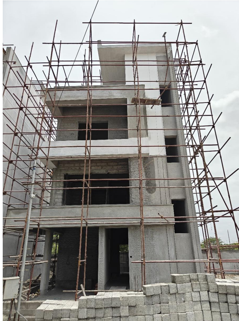
Villa No 11-Front elevation Archi concrete putty applying work in progress
