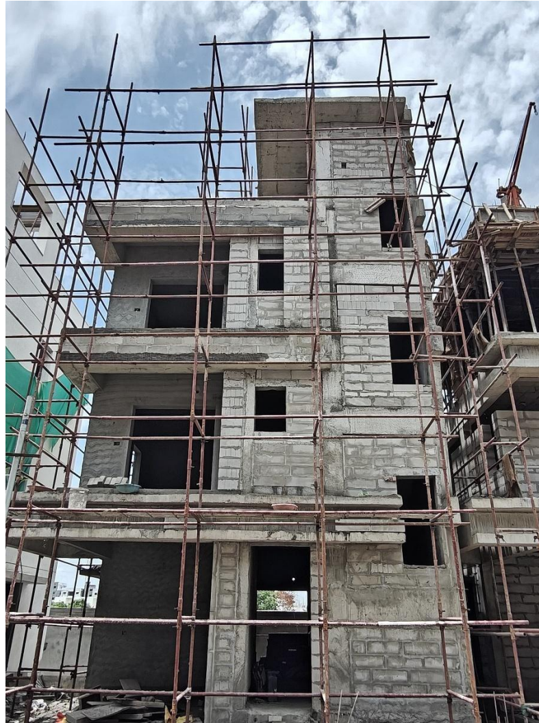
Villa No 13– Front projection slab blockwork in progress
