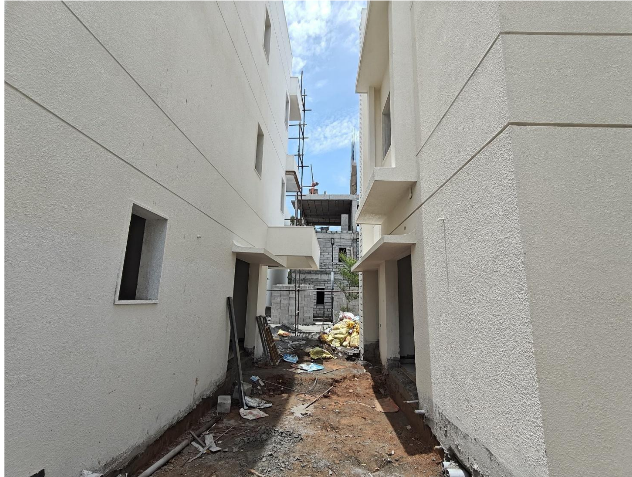
Villa No 5-6 External wall 1 st coat colour paint applying work in progress
