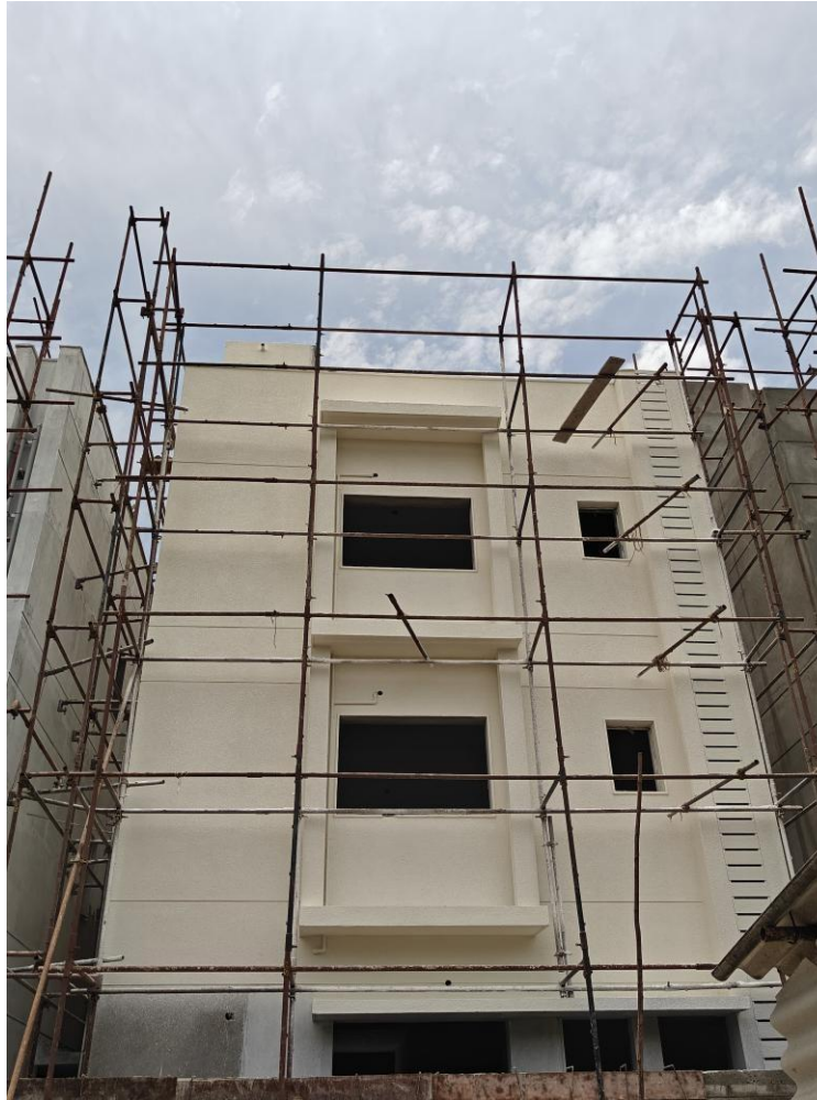
Villa No 9 – Backside elevation 1 st coat colour painting work in progress
