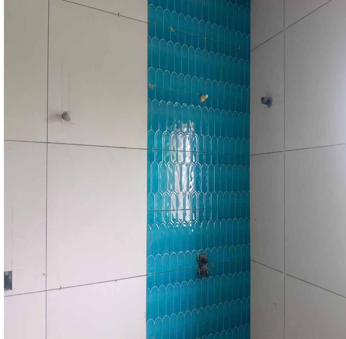
Villa No 12- FF&SF Toilet wall Laying work Completed
