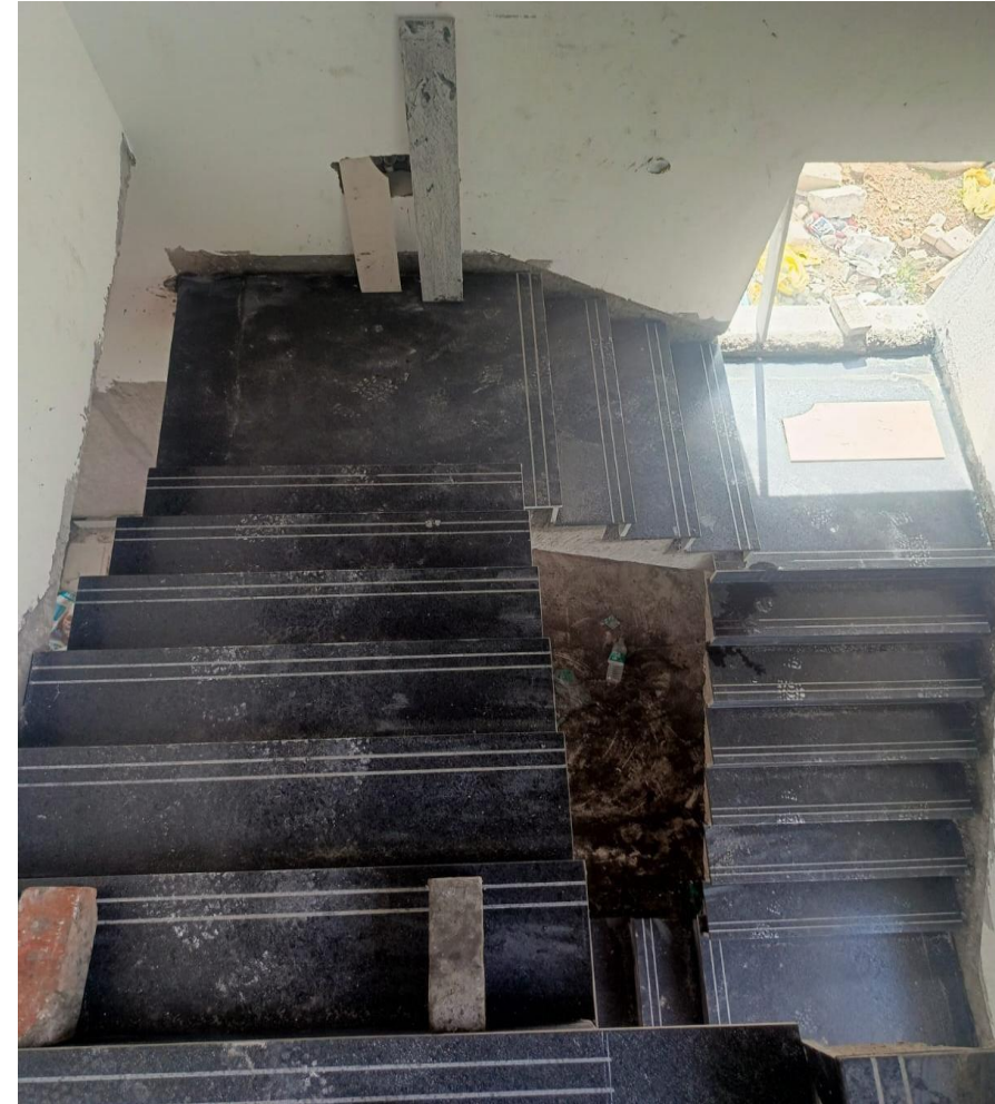
Villa No 12- Staircase Granite Laying Work Completed
