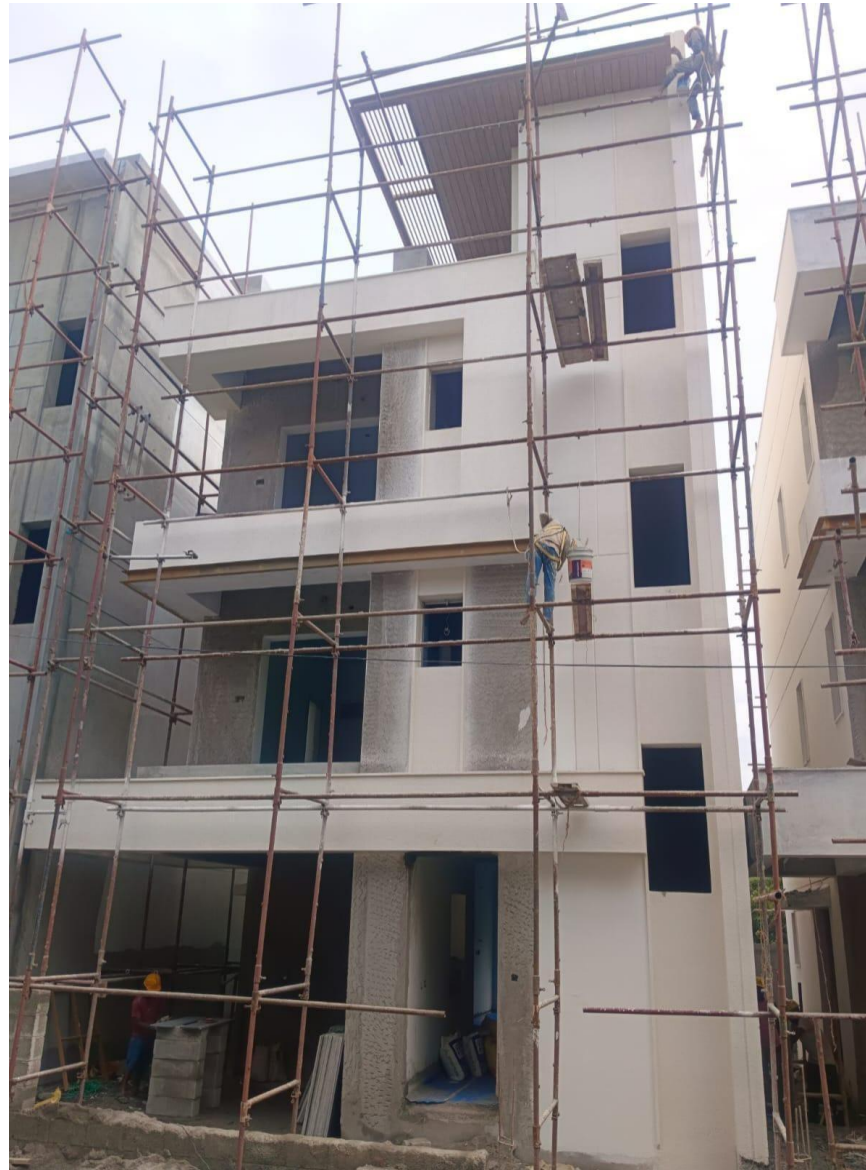
Villa No 9 –Front Elevation MS Channel Primer applying work in progress
