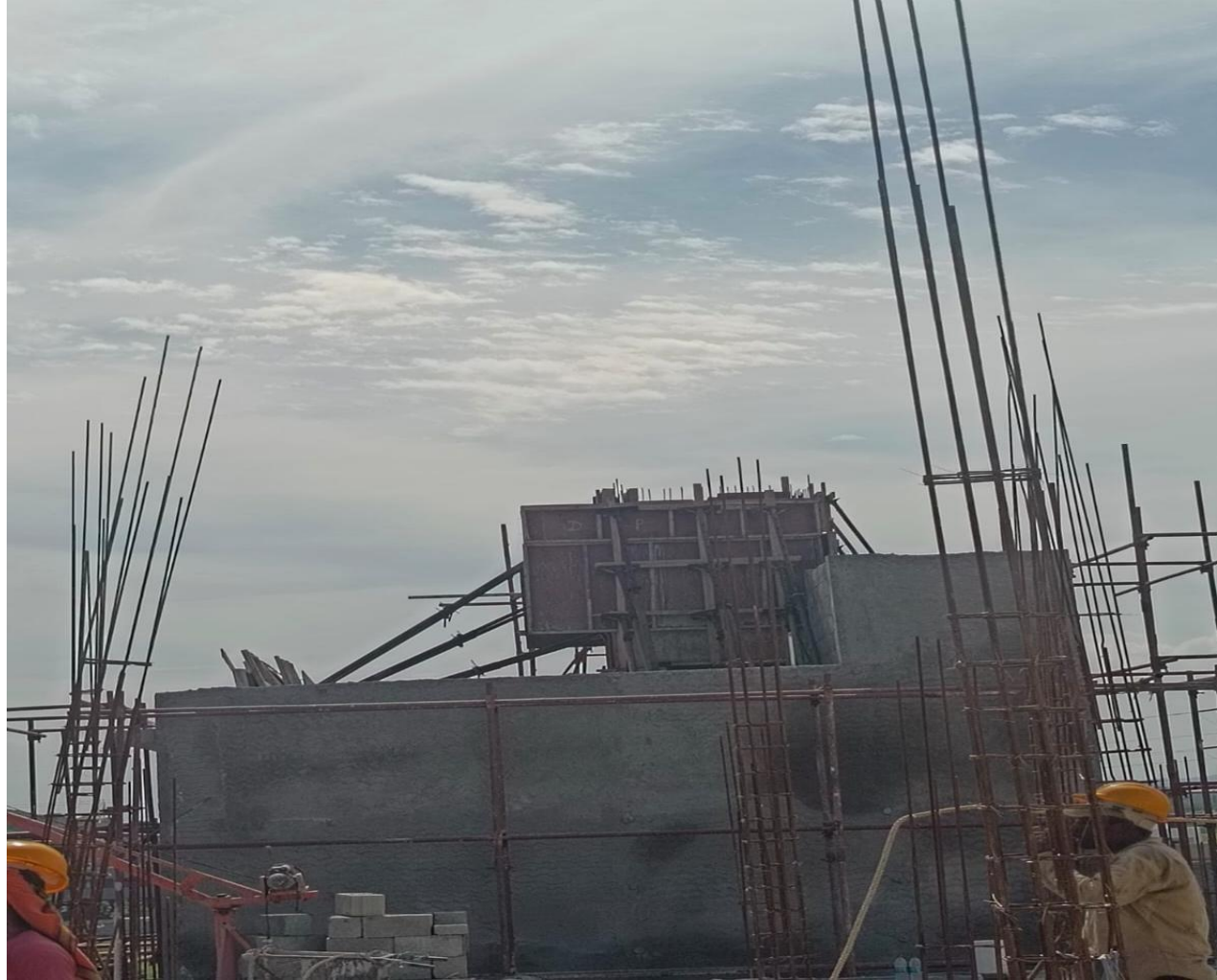
Villa No 13-OHT Tank Shuttering work in Progress
