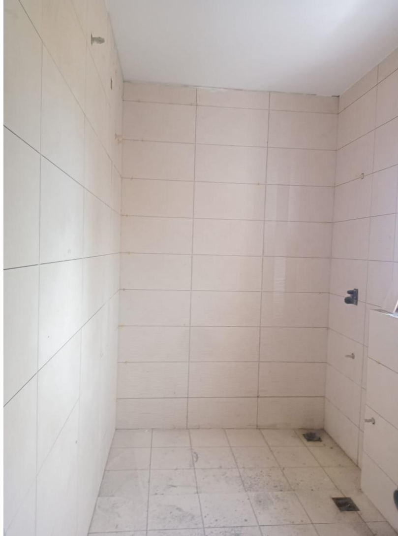
Villa No 3- FF Toilet Tile Laying work Completed
