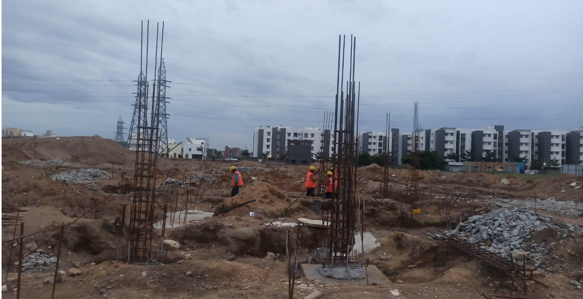
Phase 2 – villa no 53 Column Reinforcement work in progress
