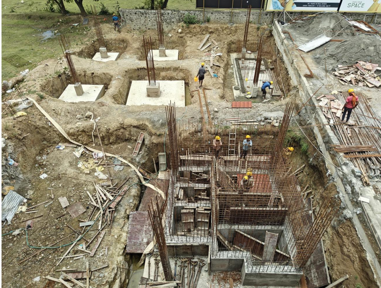
Villa No 18 – STP wall 1 st lift concreting work completed
