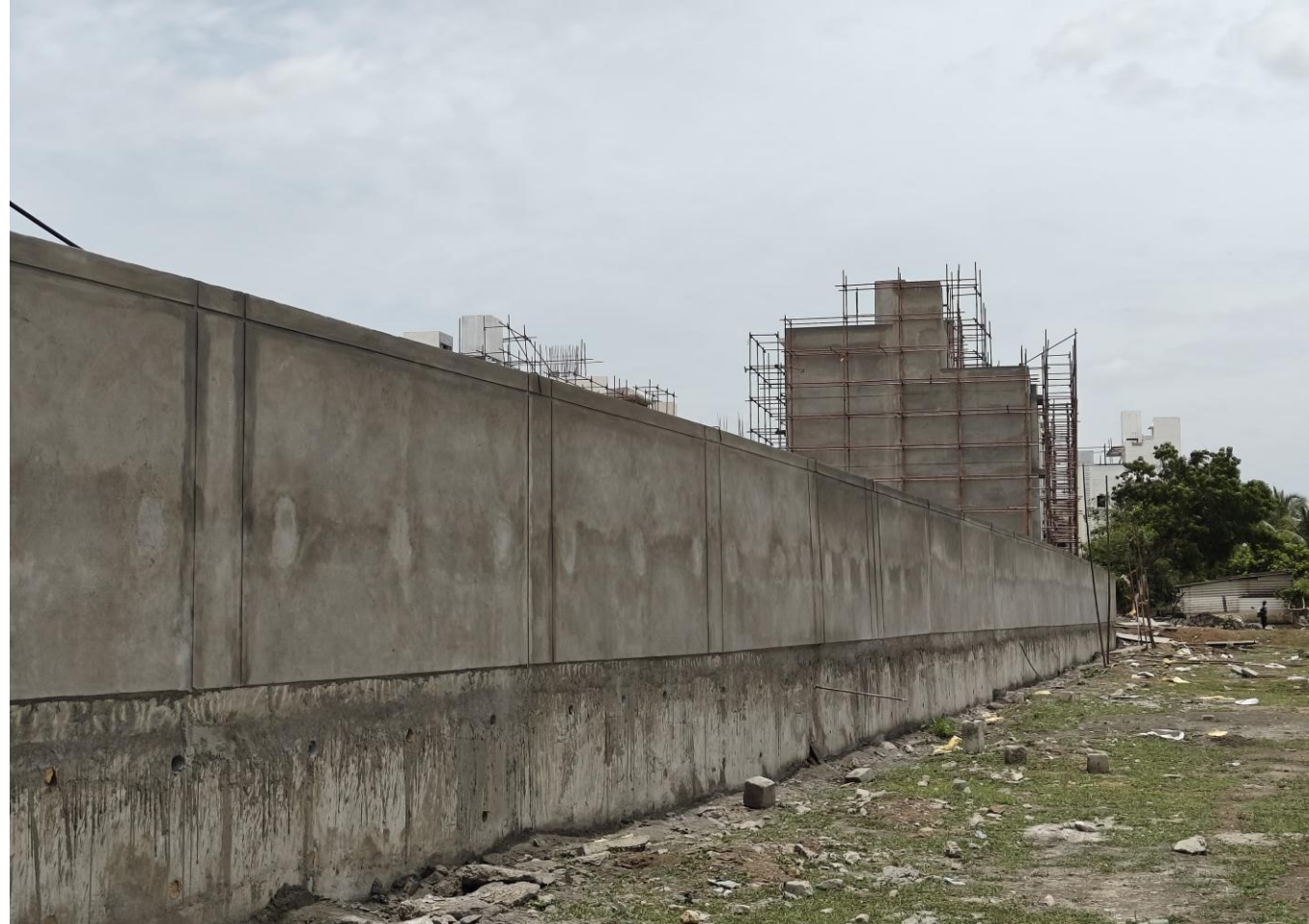
Phase 1 - Southside compound External plastering work in progress
