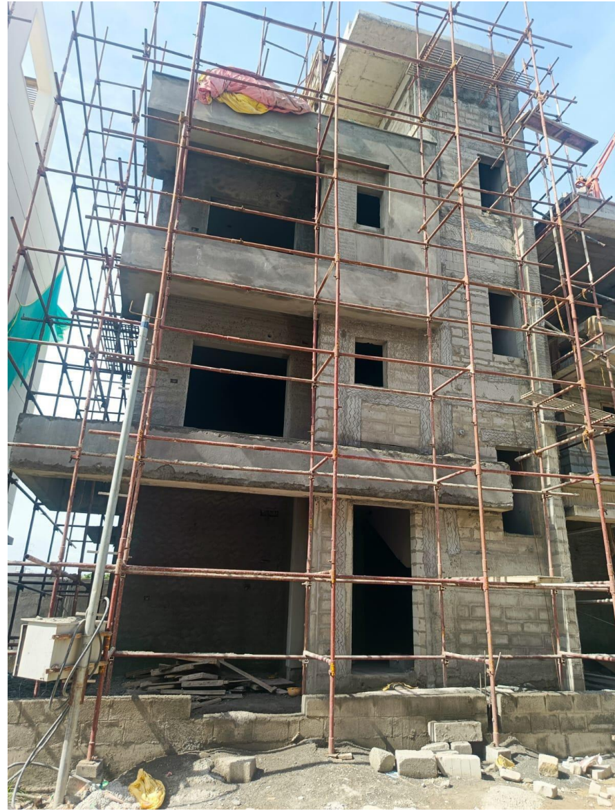
Villa No 13-Front elevation Plastering work in Progress
