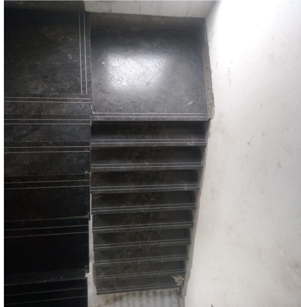
Villa No 5 Staircase Granite Laying Work Completed
