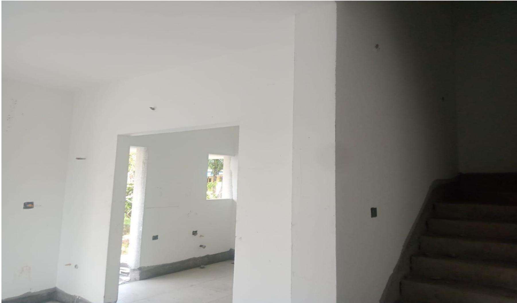
Villa No 3- WallPuttyApplying work Completed
