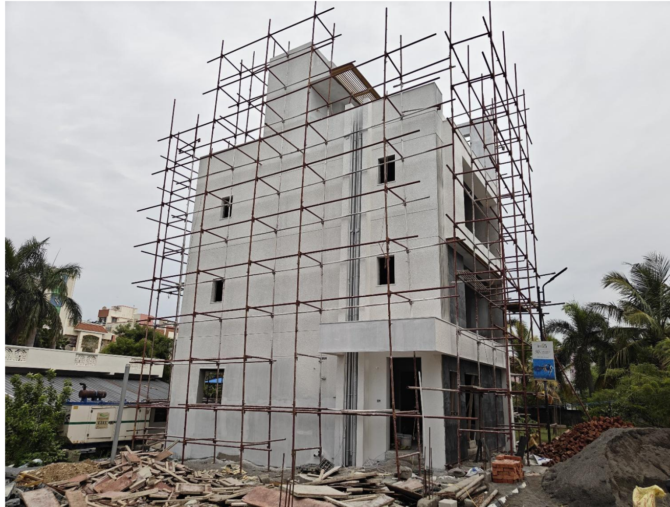
Villa No 3- Northside External wall pebble texture applying work in progress
