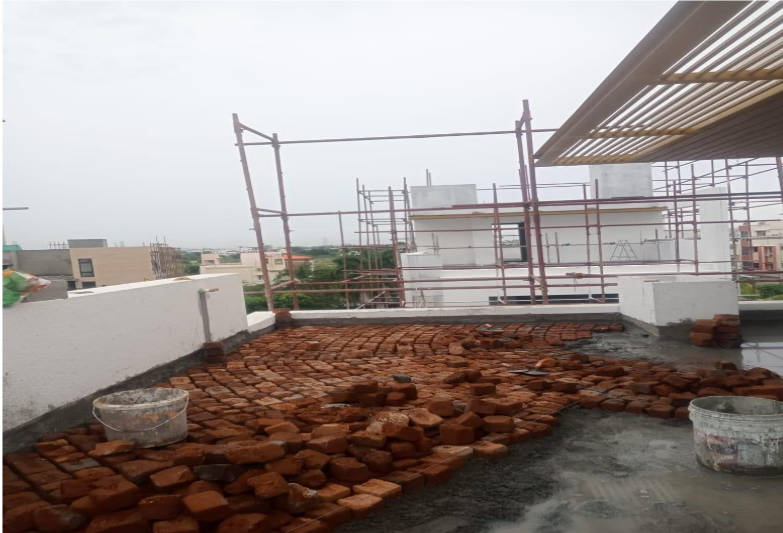
Villa No 4 – Treece Area Brick Bad Coba laying work in progress
