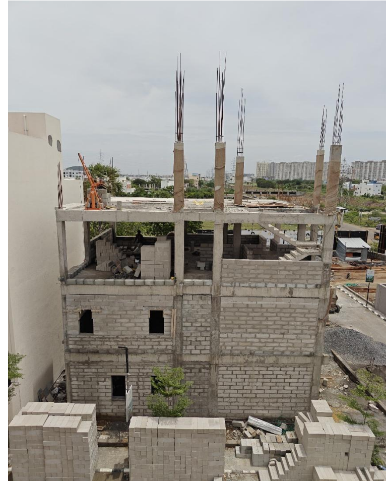
Villa No 15– Headroom column concreting work completed
