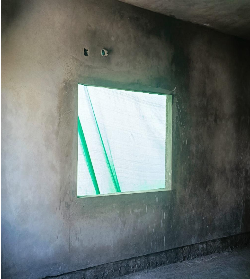
Villa No-17 FF Plastering Work In Progress
