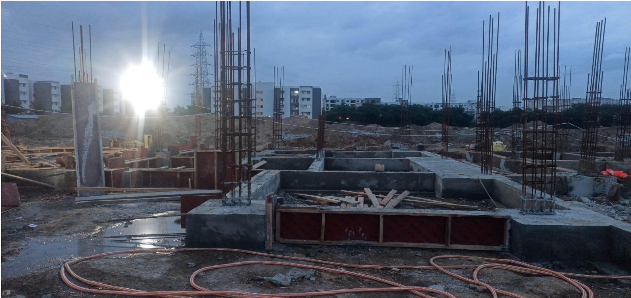
Phase 2 – villa no 49 plinth beam concrete pouring Completed
