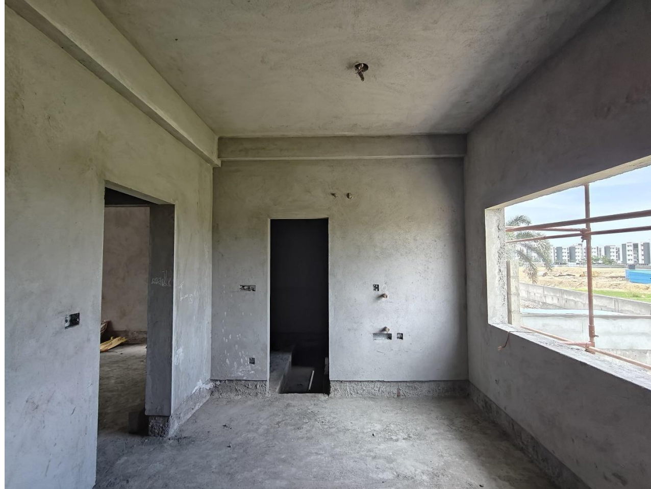
Villa No 13 – SF Bedroom Internal plastering work in progress
