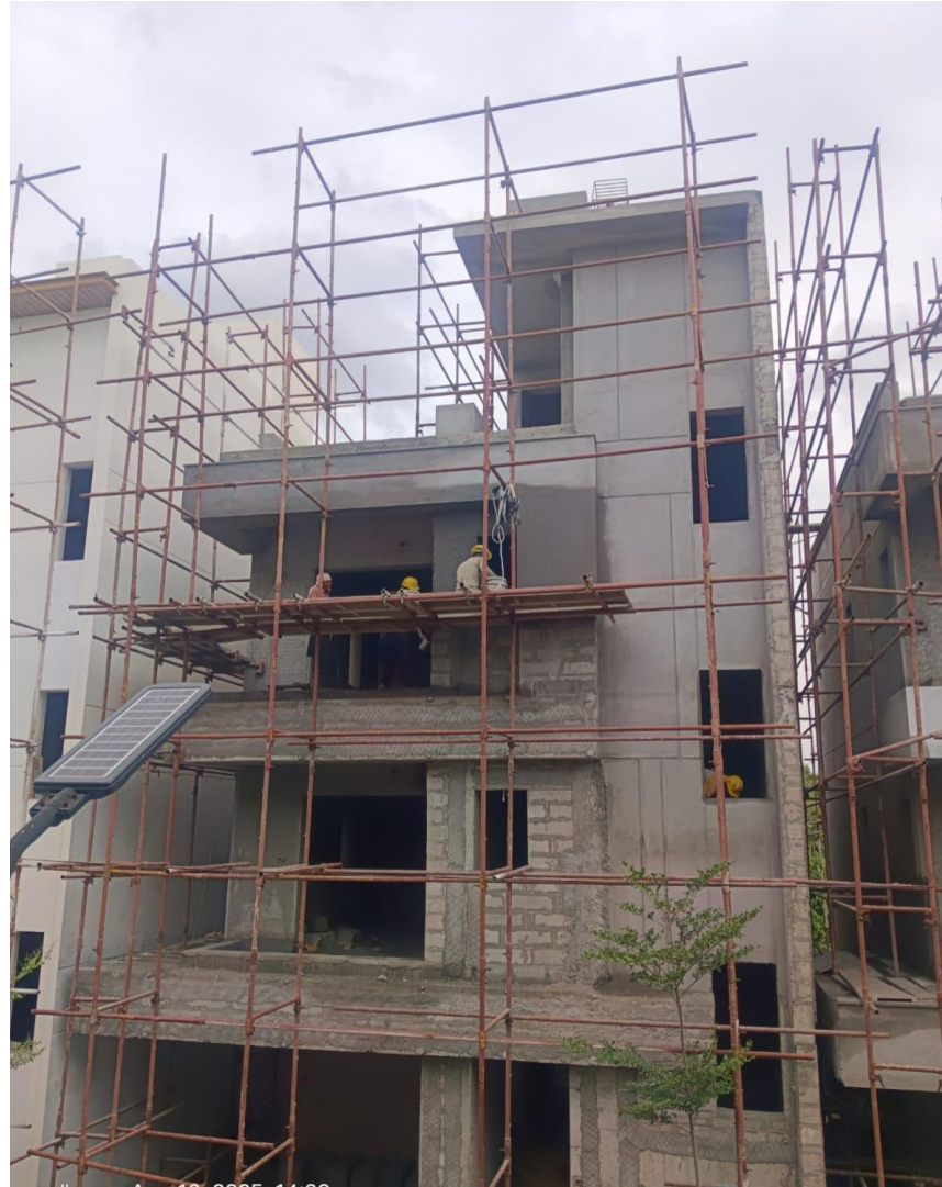
Villa No 7- Front Elevation plastering work in progress
