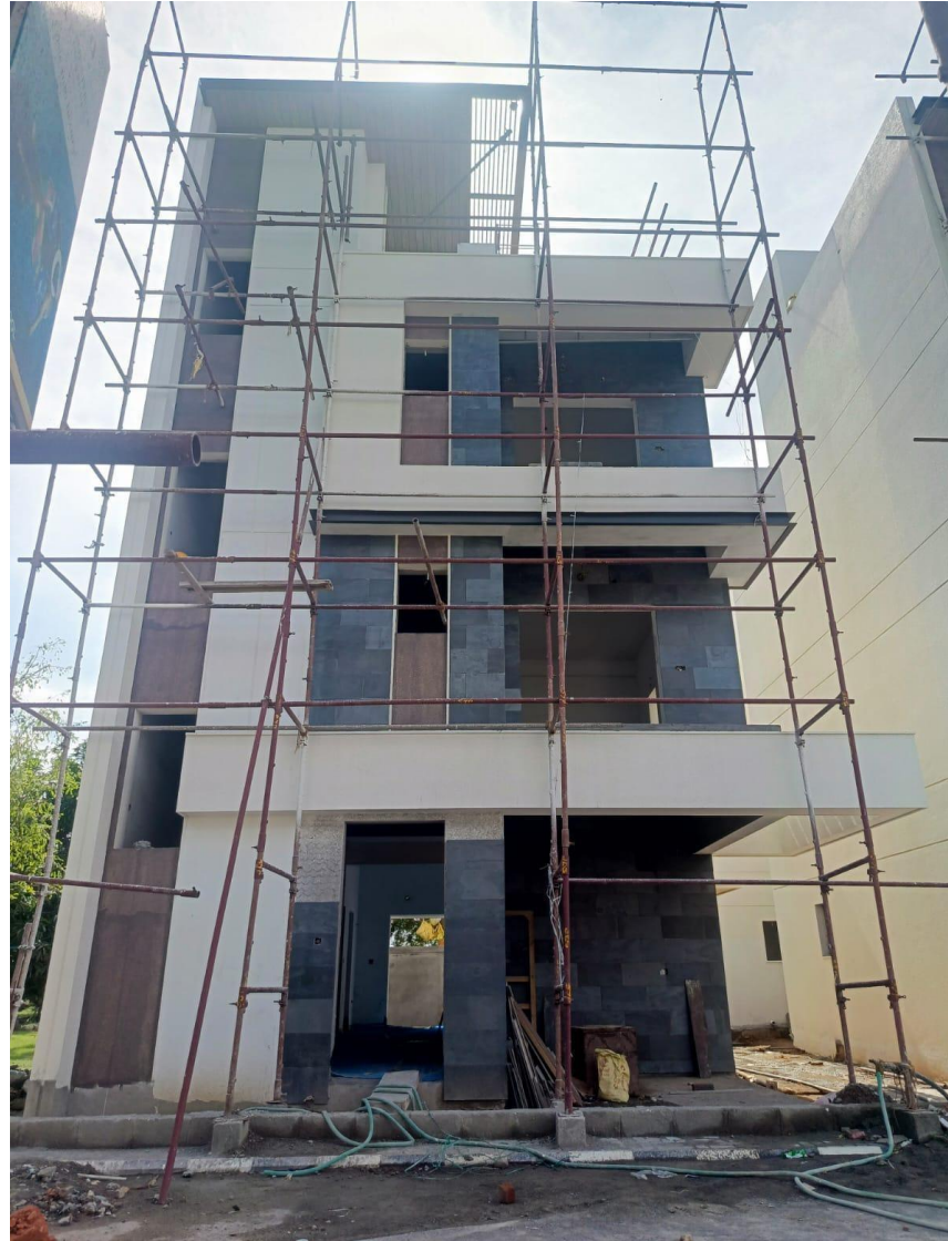
Villa No 4 – Front Elevation Staircase Painting work Completed
