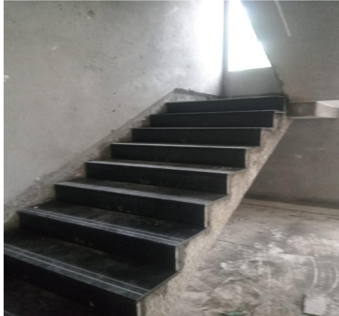
Villa No 6 Staircase Granite Laying Work Progress
