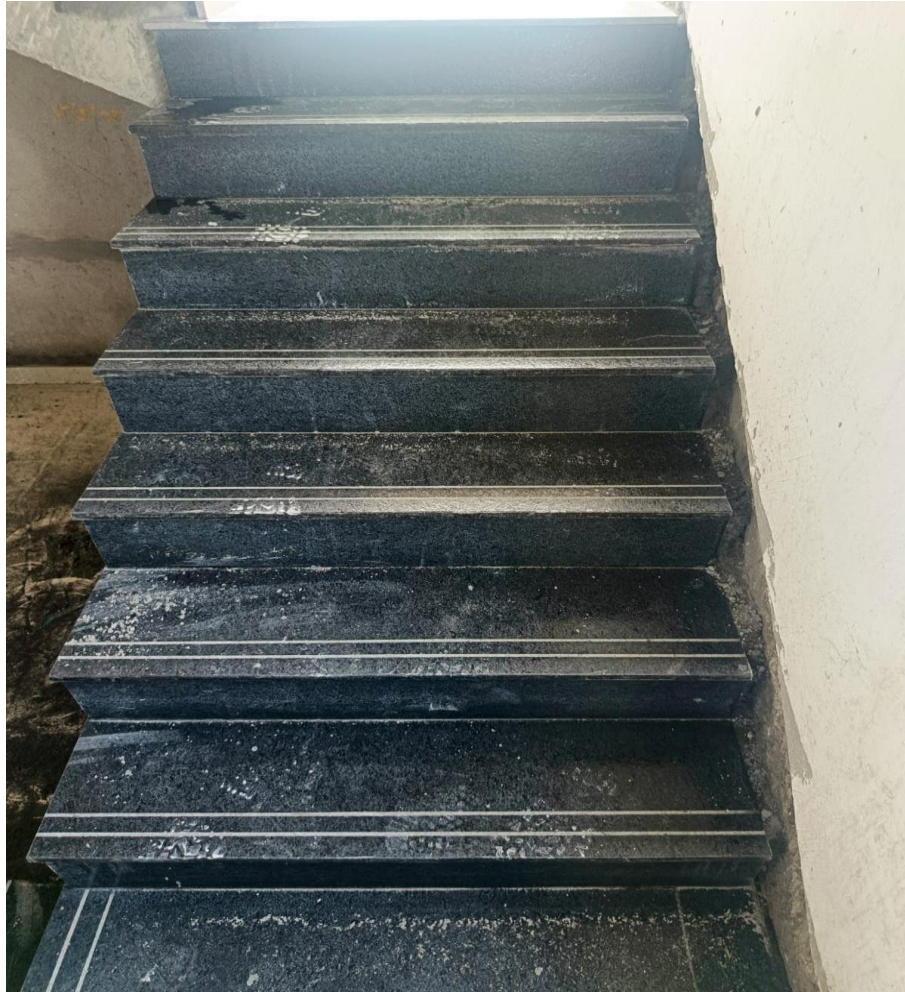
Villa No 12- Staircase Granite Laying Work Completed
