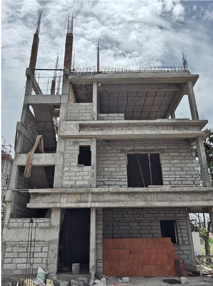
Villa No 15– Headroom column concreting work completed
