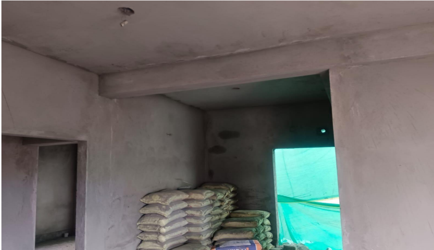
Villa No-17 GF Plastering Work Completed
