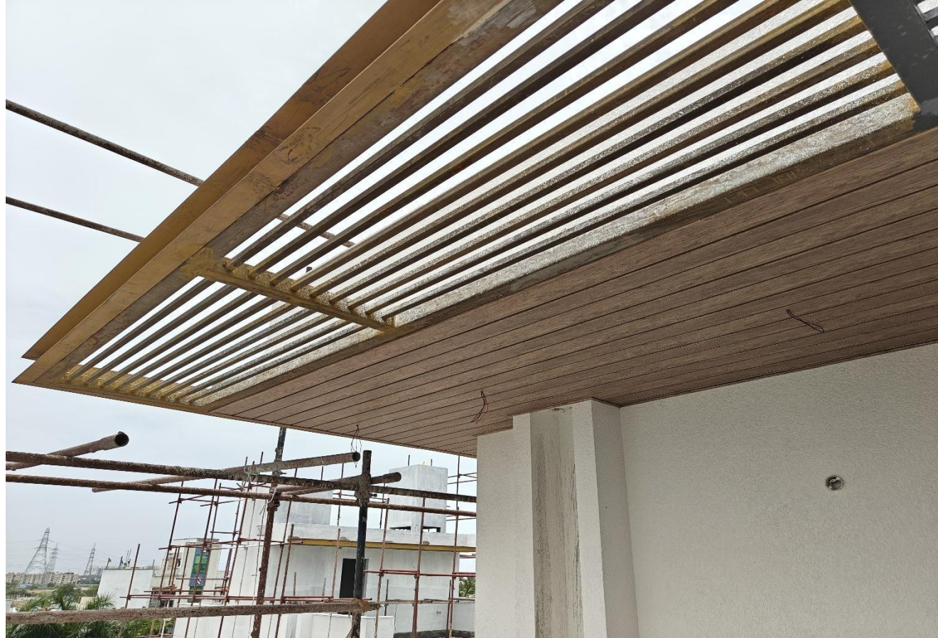
Villa No 5 – Terrace area vox false ceiling fixing work in progress
