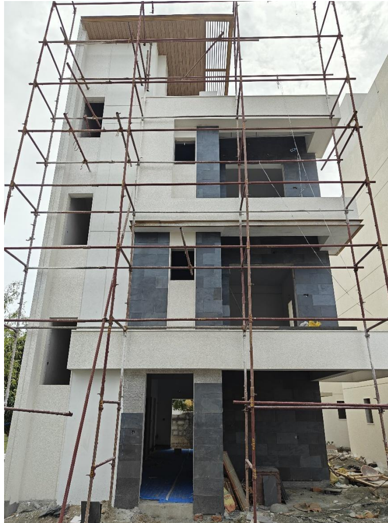
Villa No 4 – Front Elevation Slate tile laying work in progress
