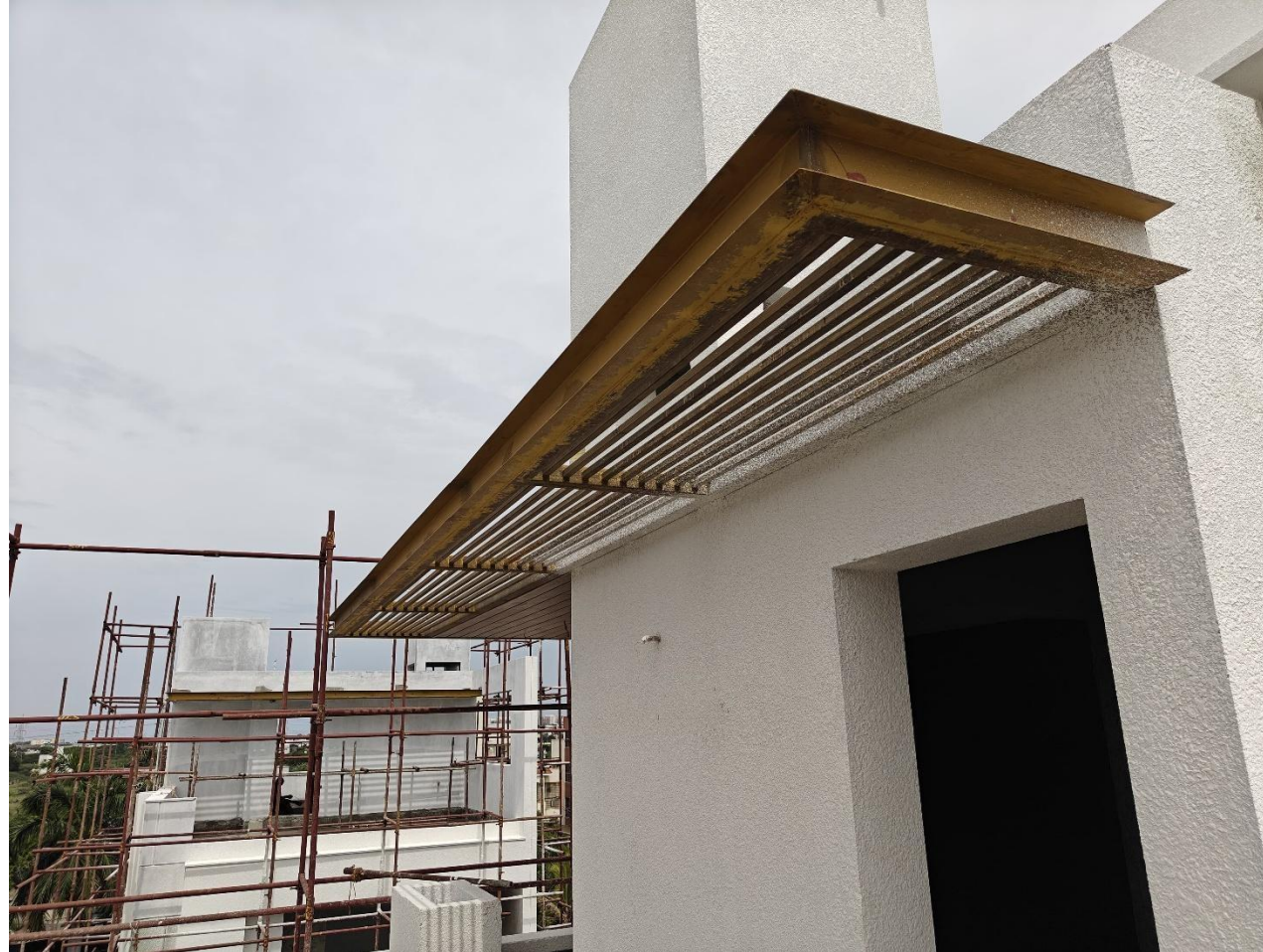
Villa No 4 – Terrace area M.S Pecola fixing work in progress
