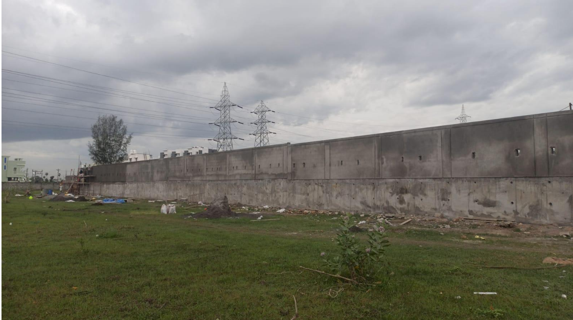
Phase 2 - Southside compound wall Plastering work in progress
