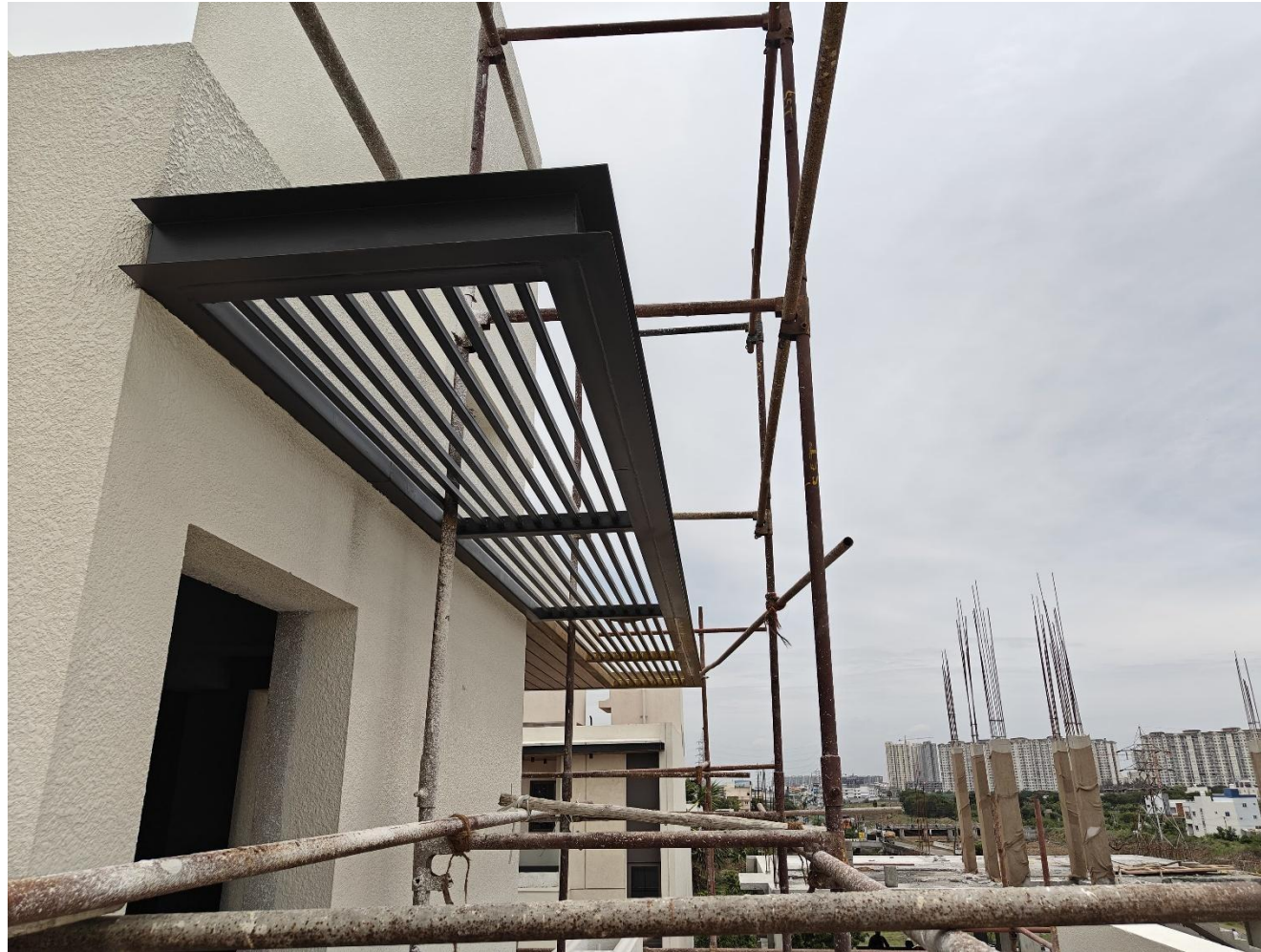
Villa No 6 – Terrace area M.S Percola enamel applying work in progress
