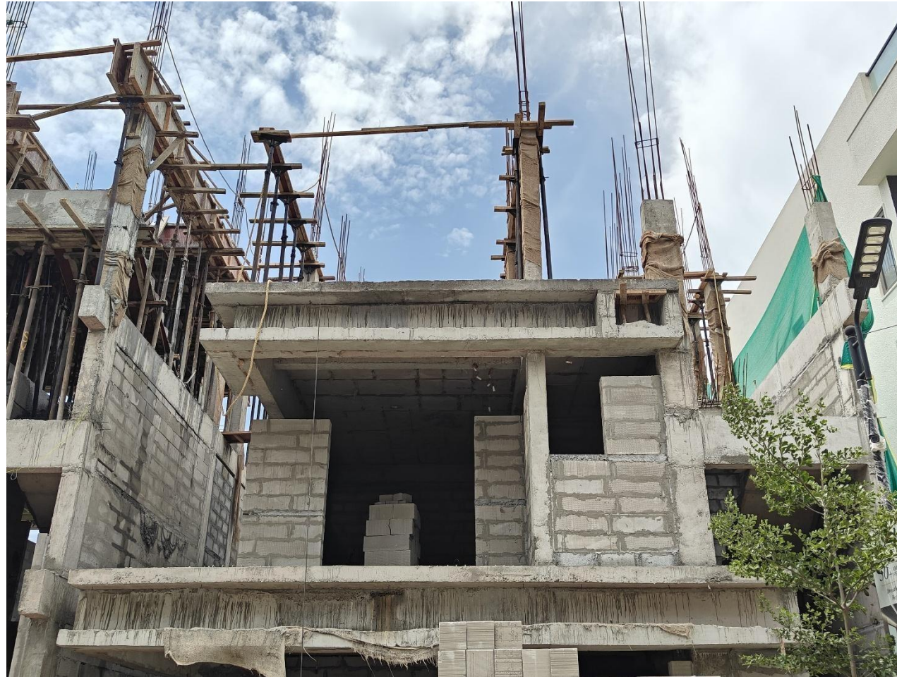
Villa No 15– SF Roof slab shuttering work in progress
