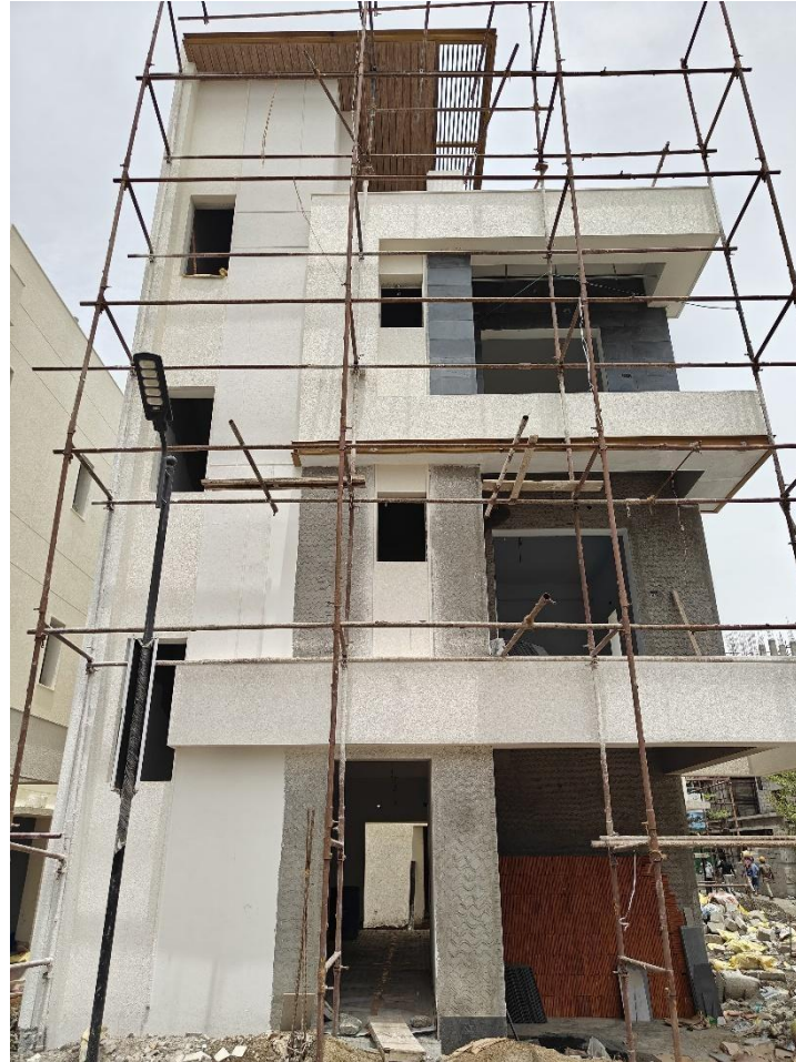
Villa No 5 – SF Balcony Elevation slate tile laying work in progress
