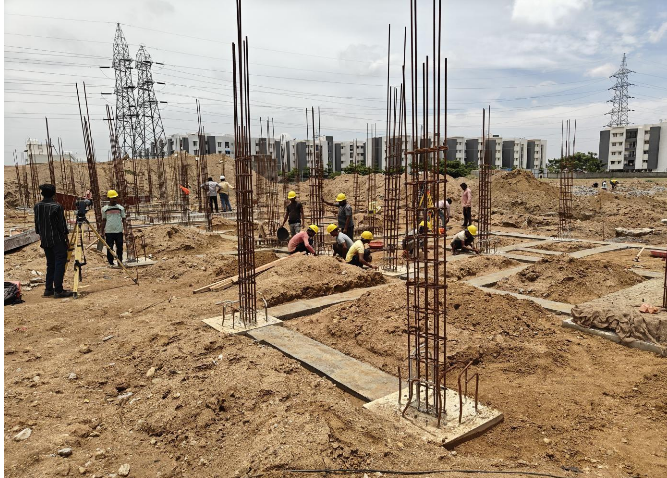
Phase 2 – villa no 50, 51 plinth beam pcc concrete pouring work in progress
