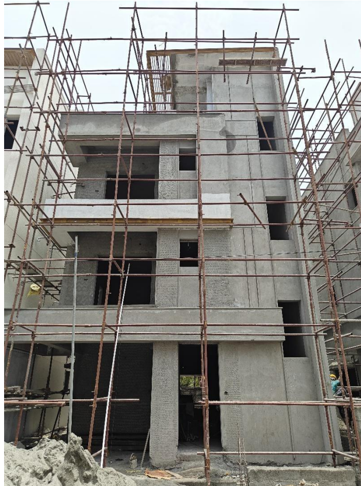
VillaNo 10- Front elevation external primer applying work in progress
