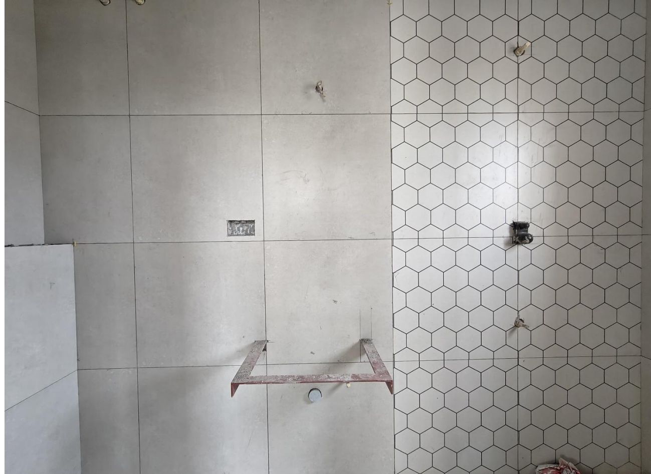
Villa No 6- FF Bedroom toilet wall tile laying work in progress
