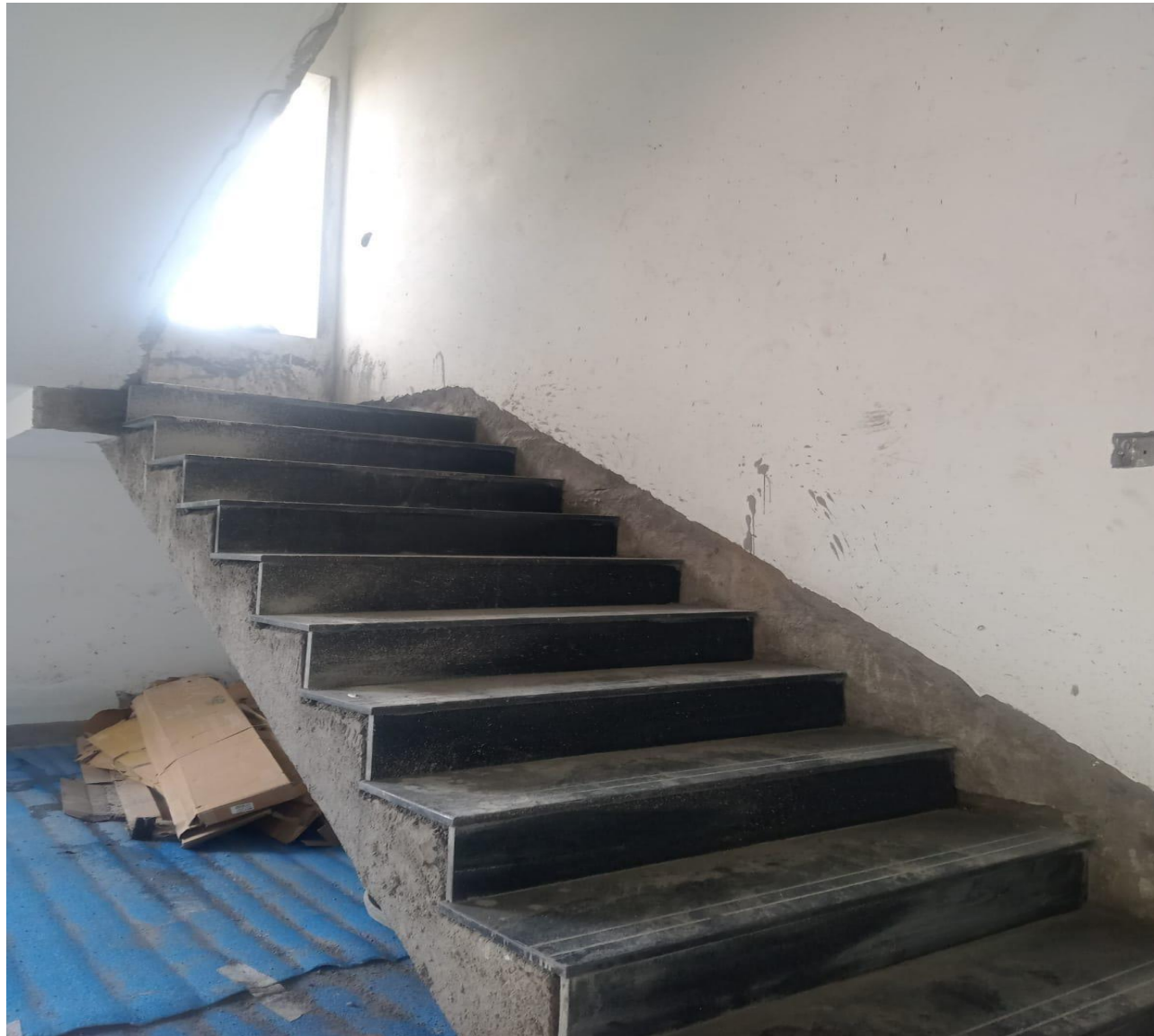
Villa No 4 – Staircase Granite Laying Work Completed
