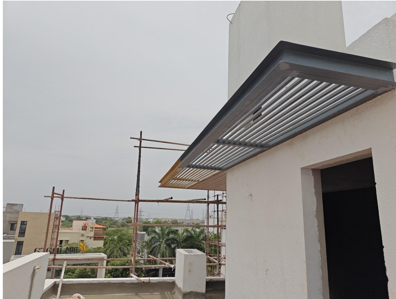
Villa No 5 – Terrace area M.S Percola enamel applying work in progress
