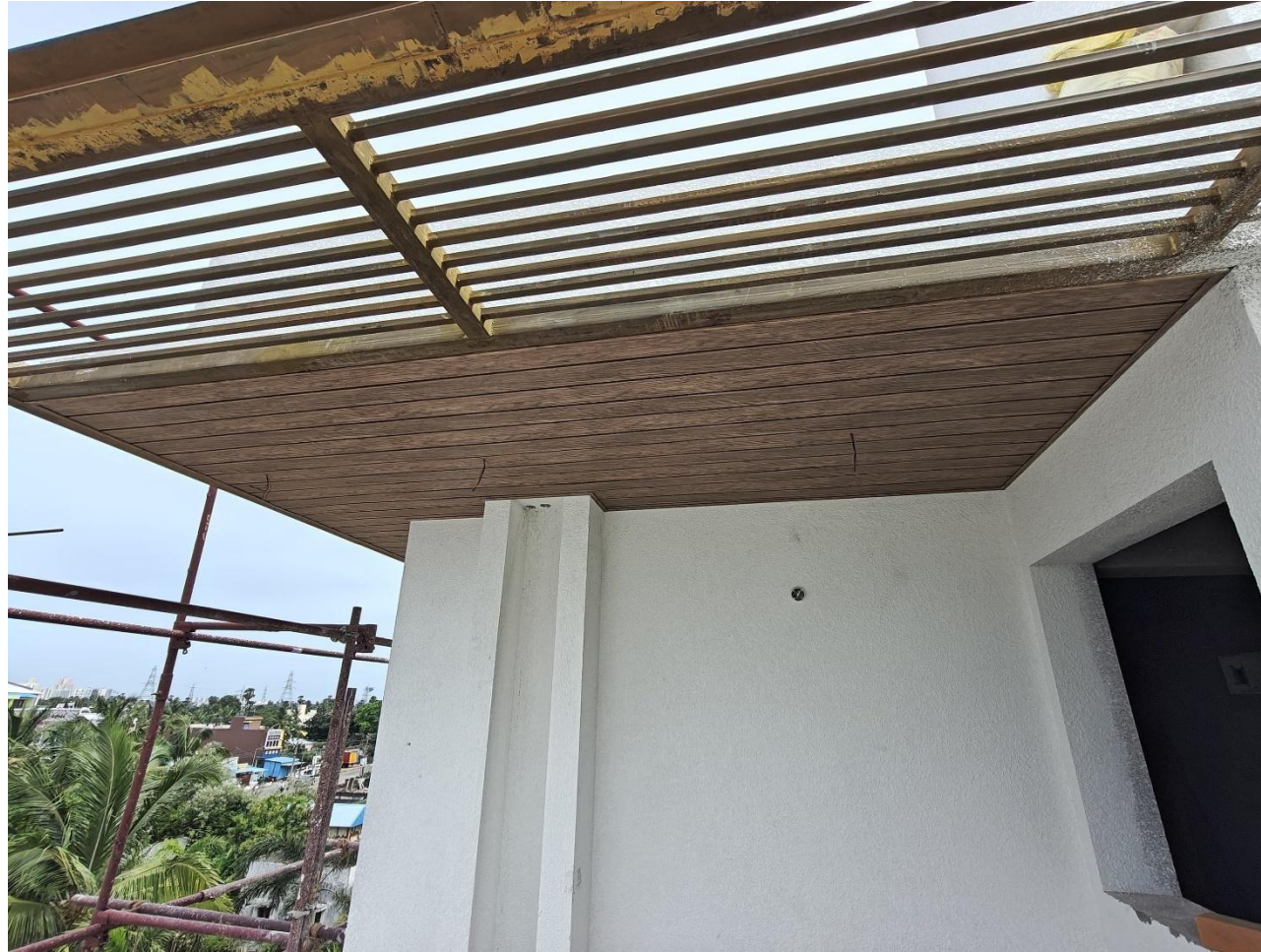
Villa No 4 – Terrace area vox false ceiling fixing work in progress
