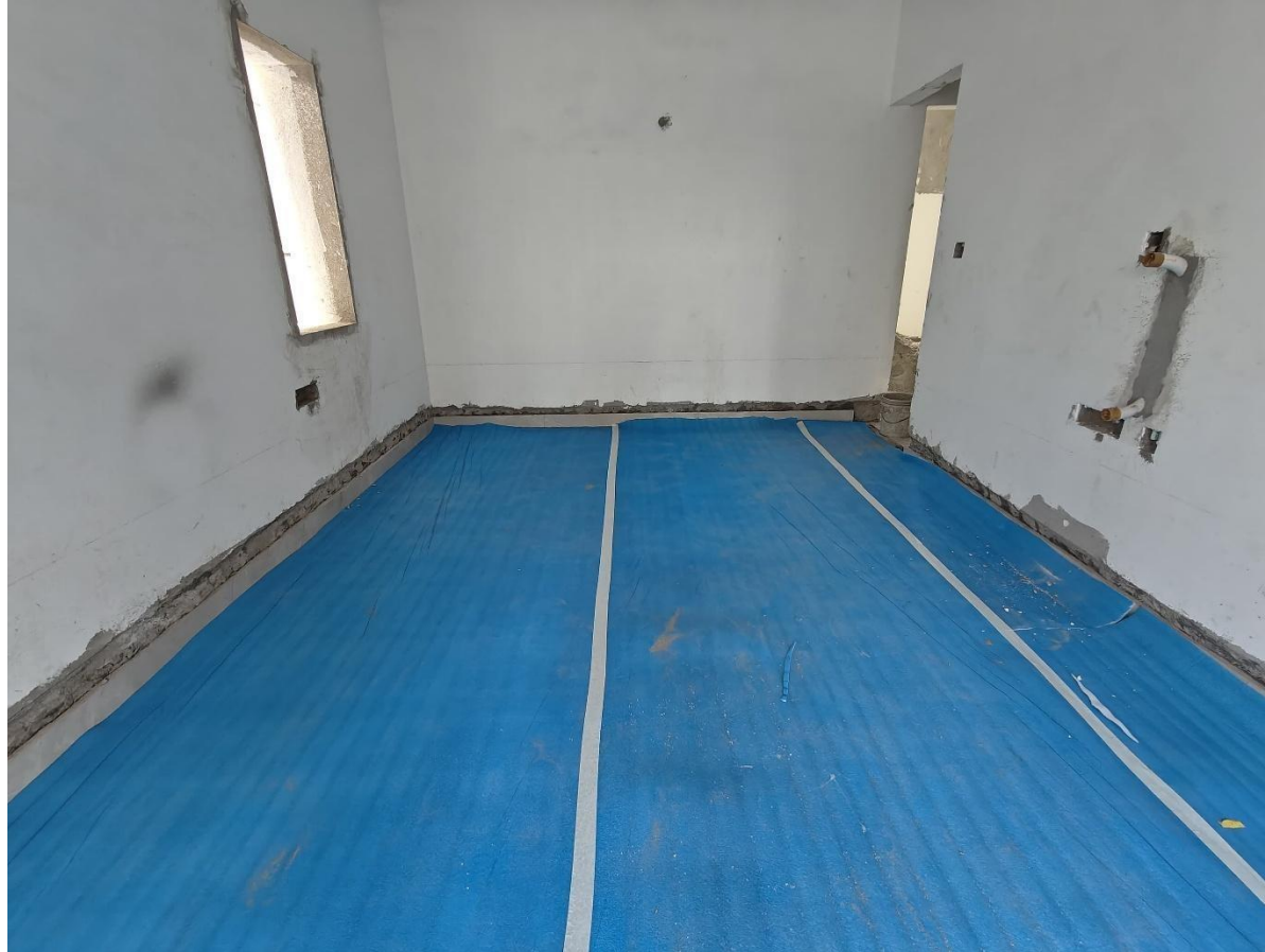
Villa No 9 – FF bedroom flooring tile protection work after tile laying
