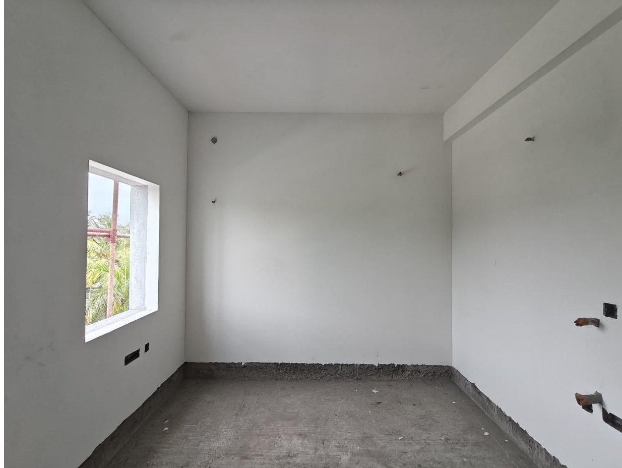
Villa No 3- SF Bedroom 1 st coat wall putty applying work in progress
