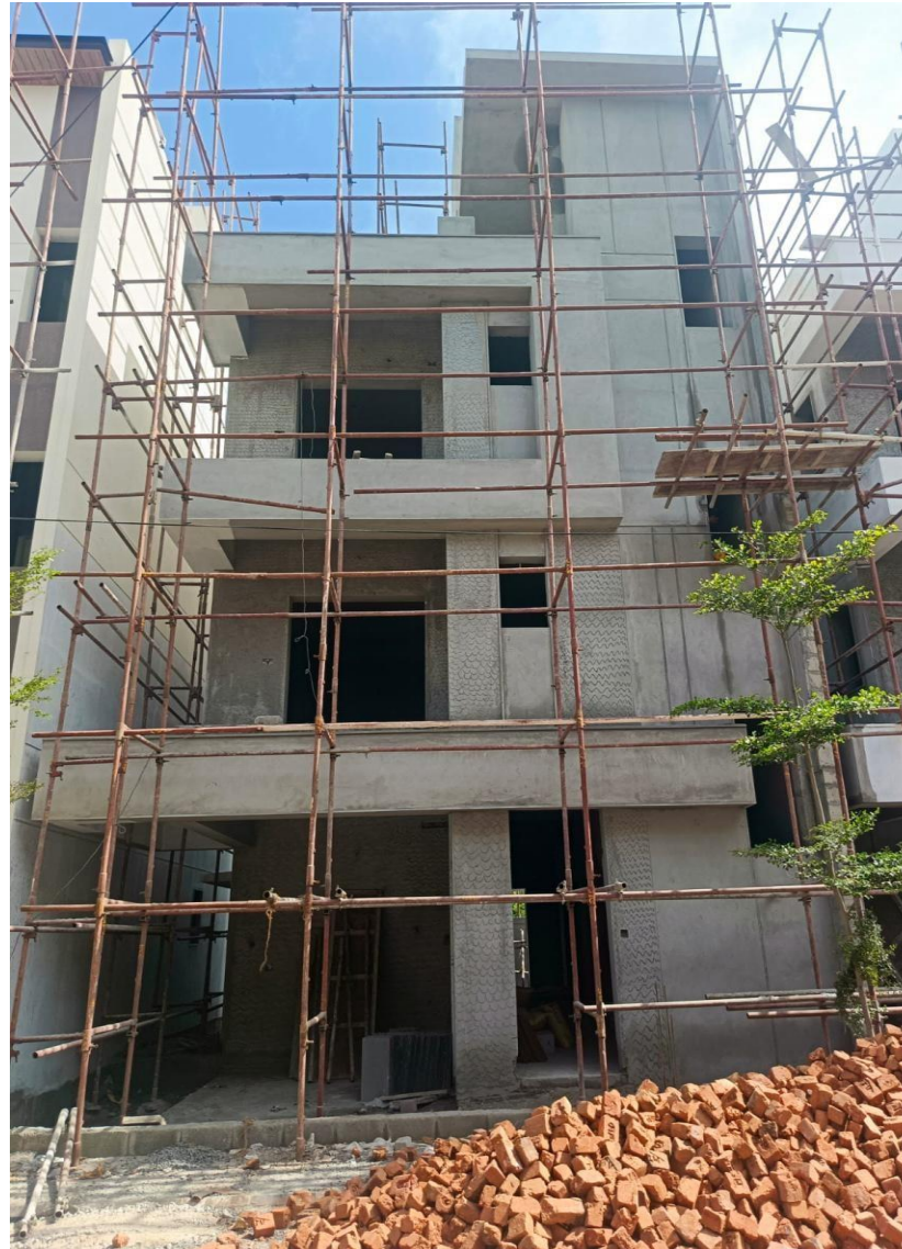
Villa No 7- Front Elevation plastering work Completed
