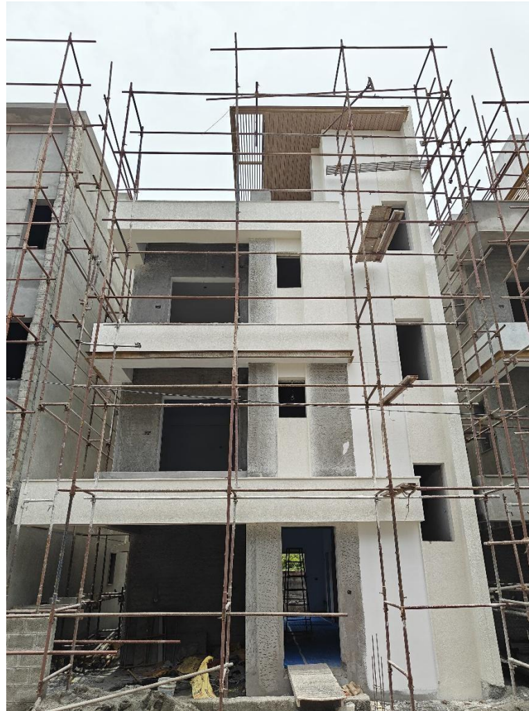
Villa No 9 –Front Elevation pebble texture applying work in progress
