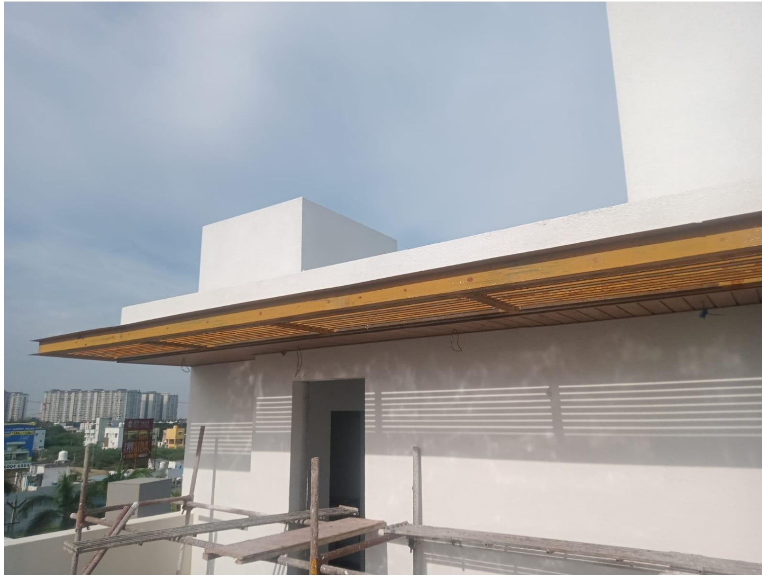
Villa No 3- MSPergolaFalseceiling work Completed
