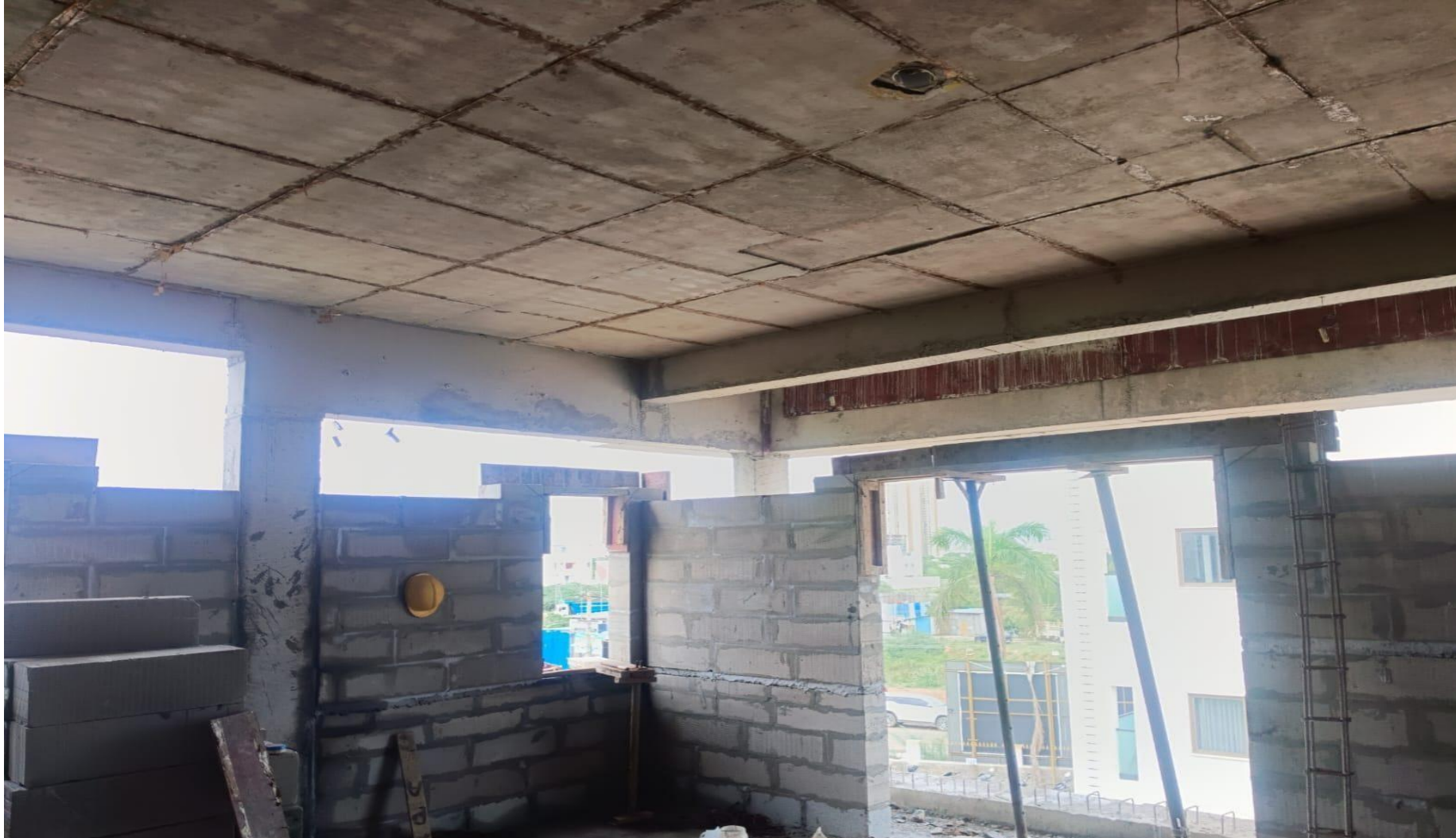
Villa No-17 SF Block Work In Progress
