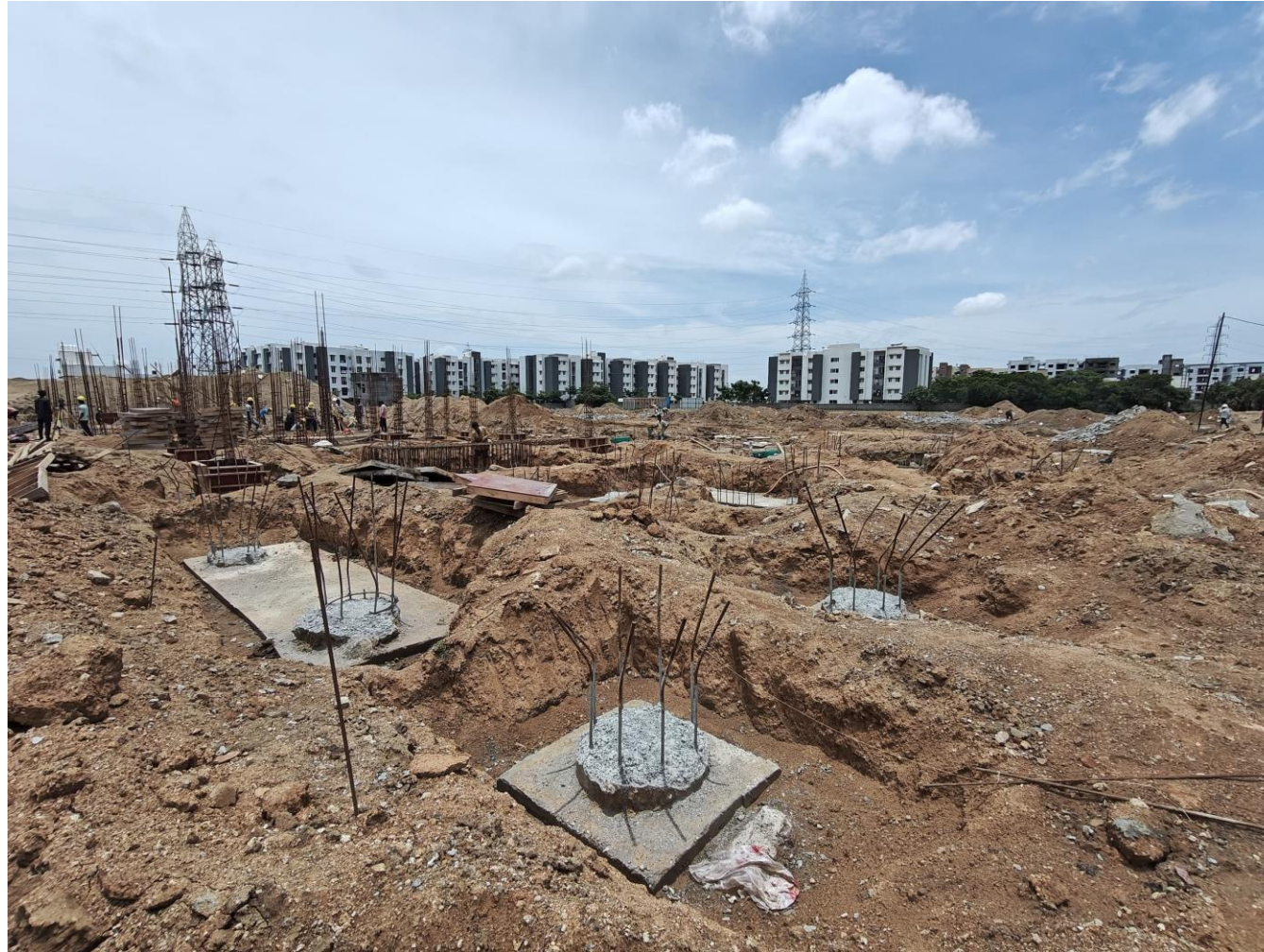
Phase 2 – villa no 53 pile cap pcc concrete pouring work in progress
