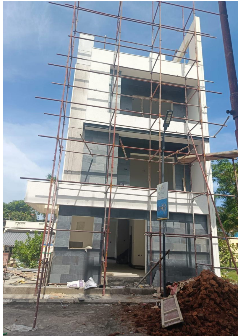
Villa No 3 – Front Elevation Slate tile laying work Completed
