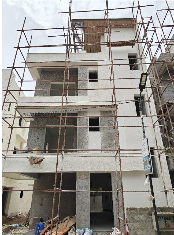
Villa No 6- Front elevation wall pebble texture applying work in progress
