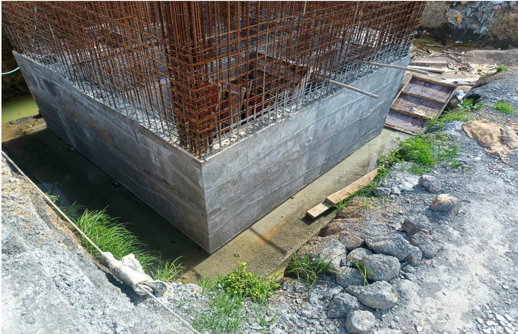
Villa No 18 – STP wall External Area Waterproofing work completed
