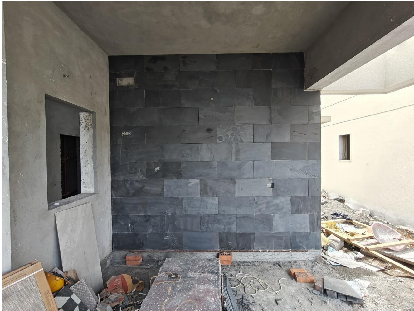
Villa No 4 – Car parking area Slate tile laying work in progress
