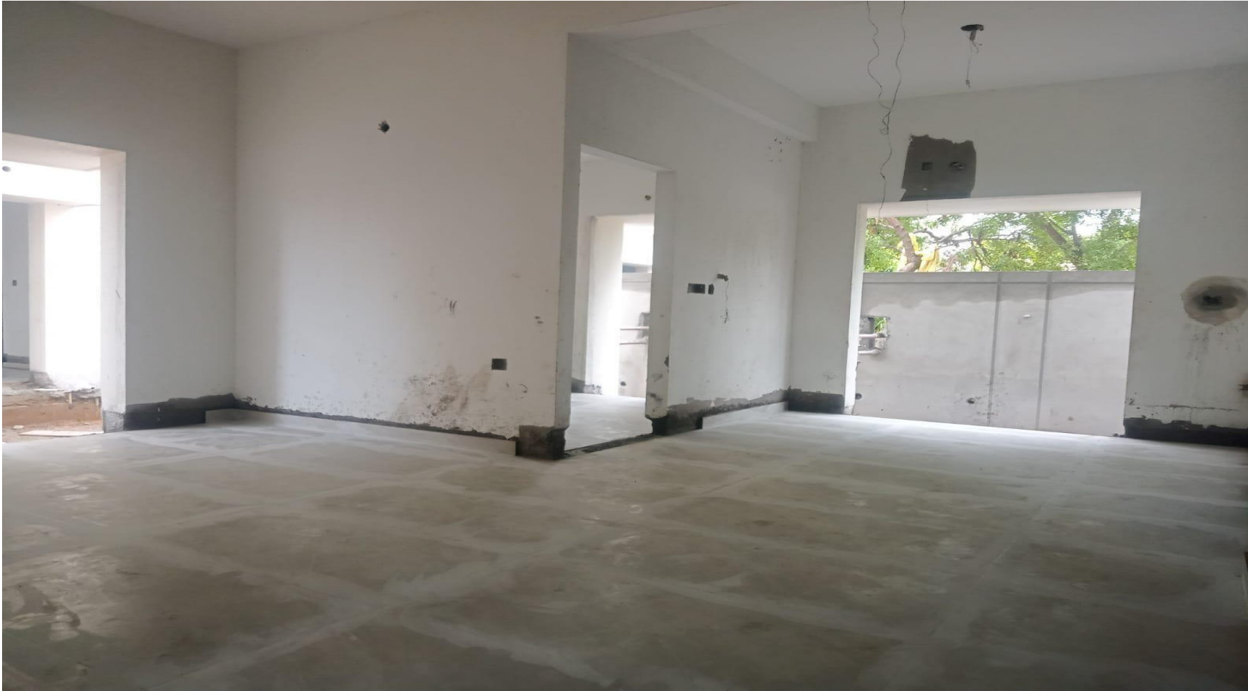
VillaNo 6 GF Flooring Tiles Laying Work Completed
