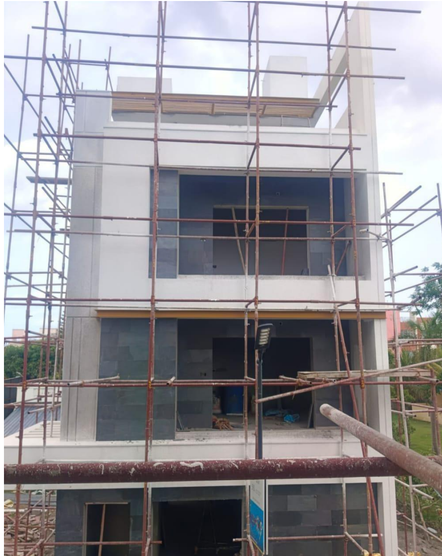
Villa No 3 – Front Elevation Slate tile laying work Completed
