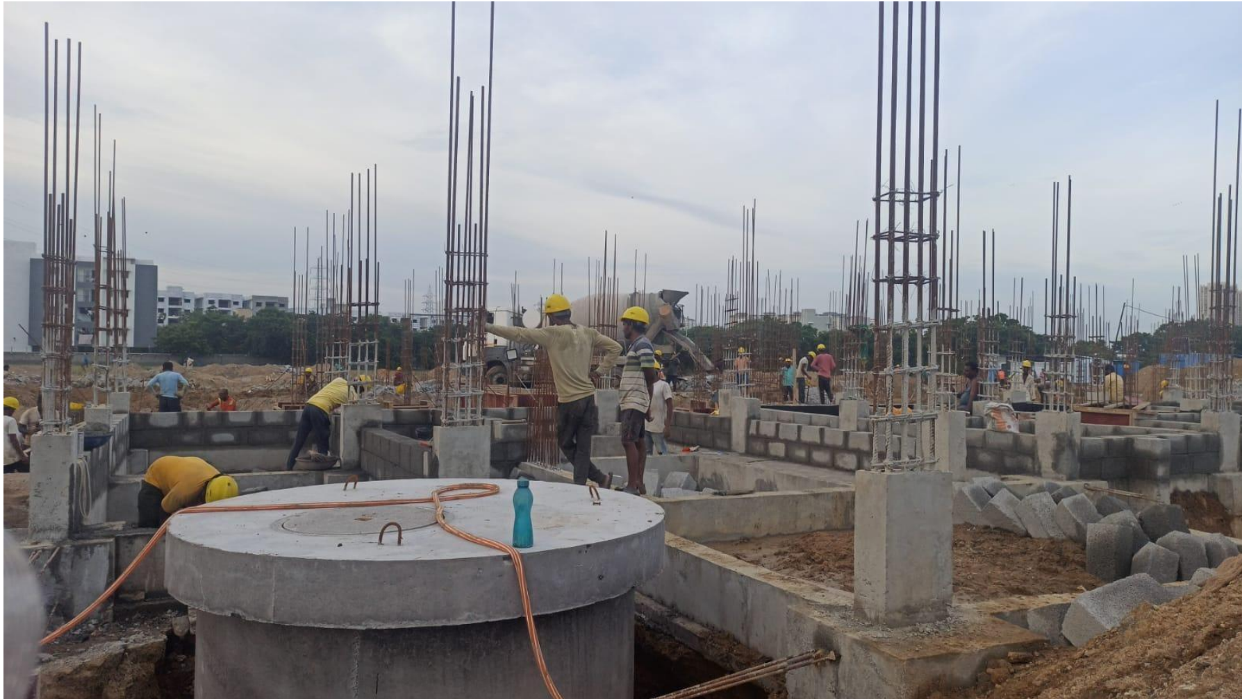
Phase 2 – villa no 49 Basement Block Work Progress
