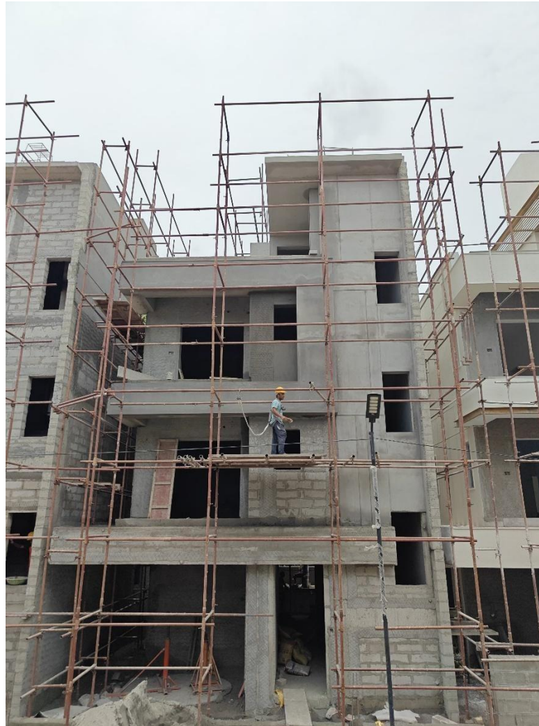
Villa No 8- Front elevation wall plastering work in progress
