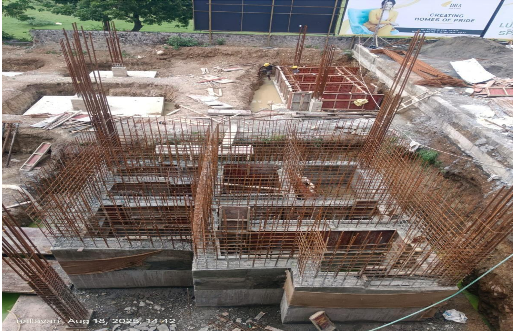
Villa No 18 – STP wall 2 nd lift concreting work completed
