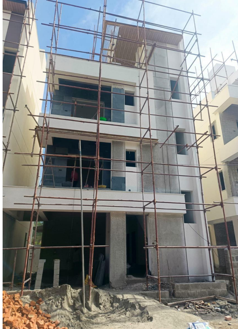
Villa No 10 –Front Elevation Slate Tiles Laying work in progress
