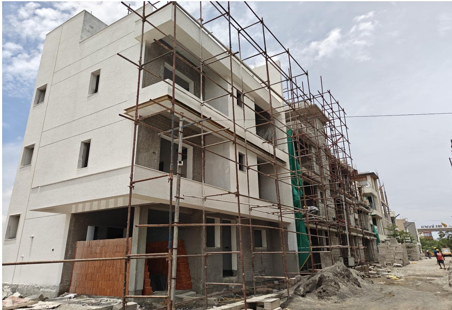
Villa No 12 – External wall pebble texture applying work in progress
