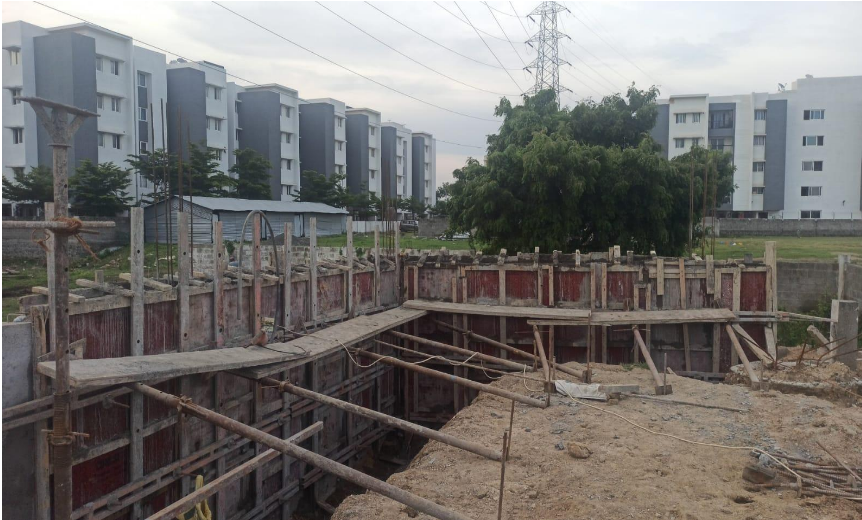
Phase 2 – North West compound wall Shuttering & Concrete pouring in Progress
