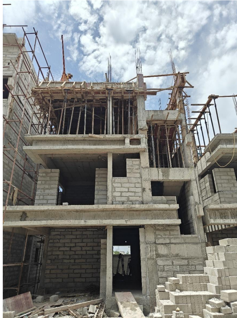
Villa No 14– SF Roof slab concreting work completed
