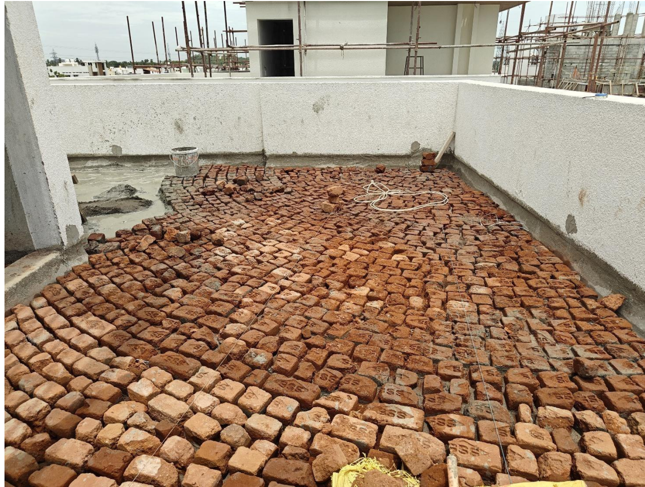
Villa No 5 – Terrace area Brickbat Cob laying work in progress
