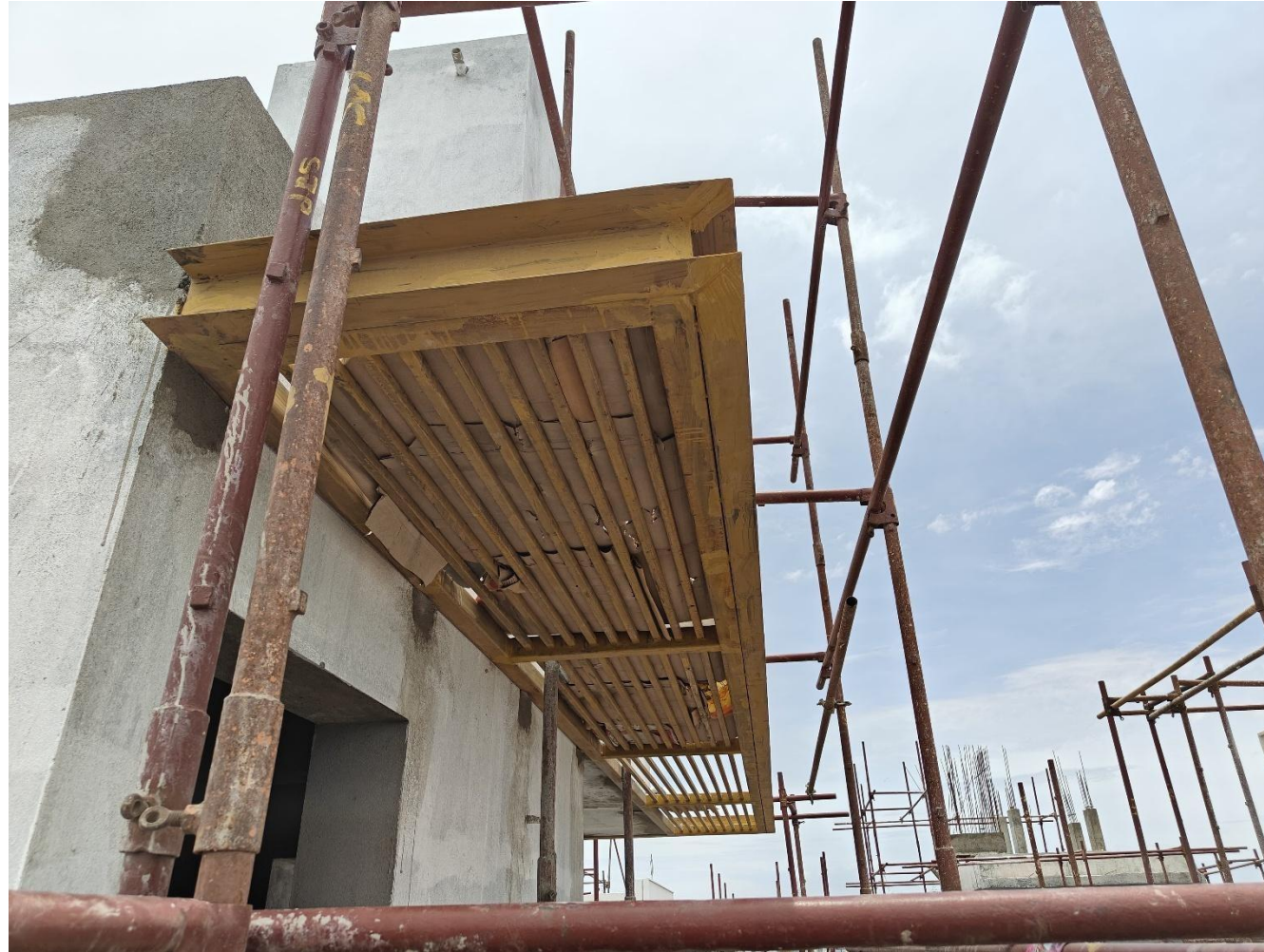
VillaNo 10- Terrace area M.S Percola fixing work in progress
