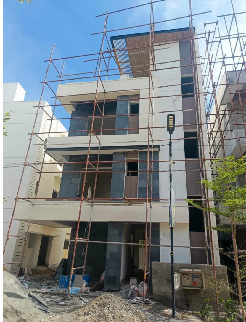
Villa No 6- Front elevation Slate Tiles Laying Work Completed
