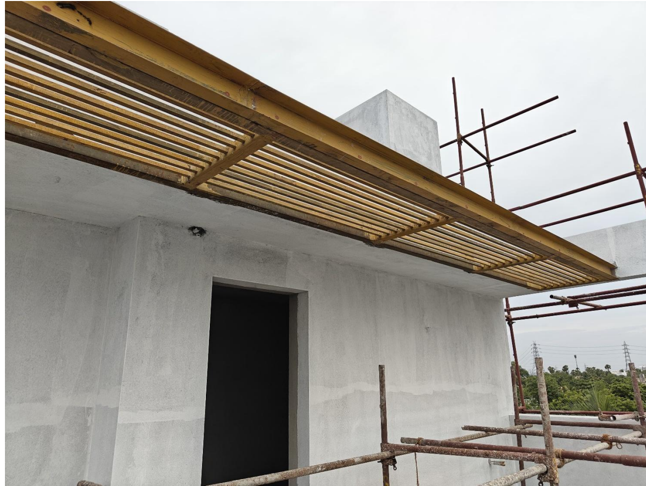
Villa No 3- Terrace area M.S Percola fixing work in progress
