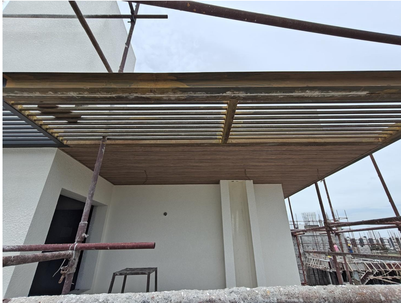
Villa No 6 – Terrace area vox false ceiling fixing work in progress
