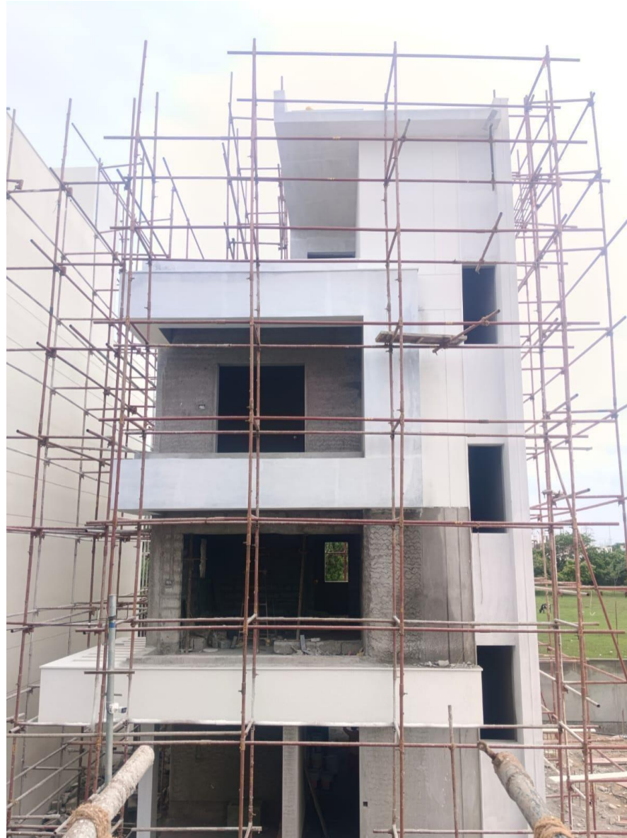
Villa No 11-Front elevation primer applying work in Completed
