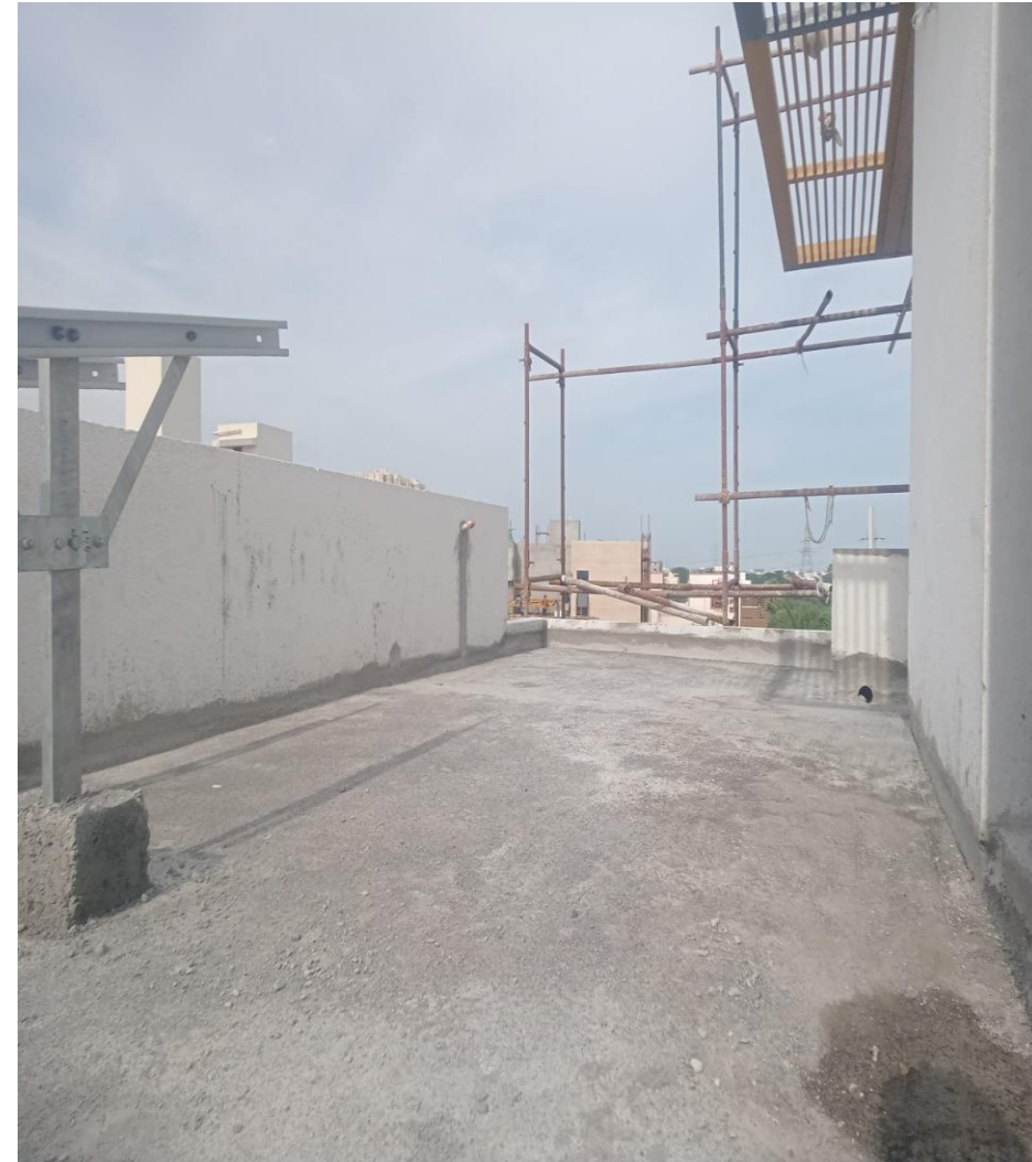
Villa No 5 ; Tracee Screed Concrete Completed
