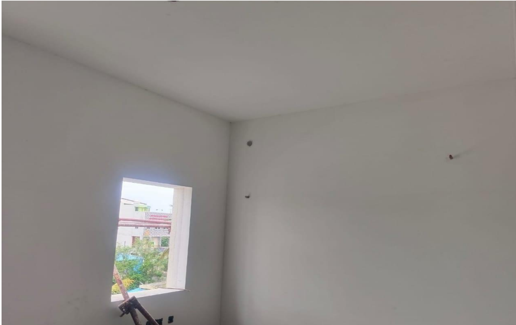
Villa No 3- SFBedRoomWallPuttyApplyingworkin progress
