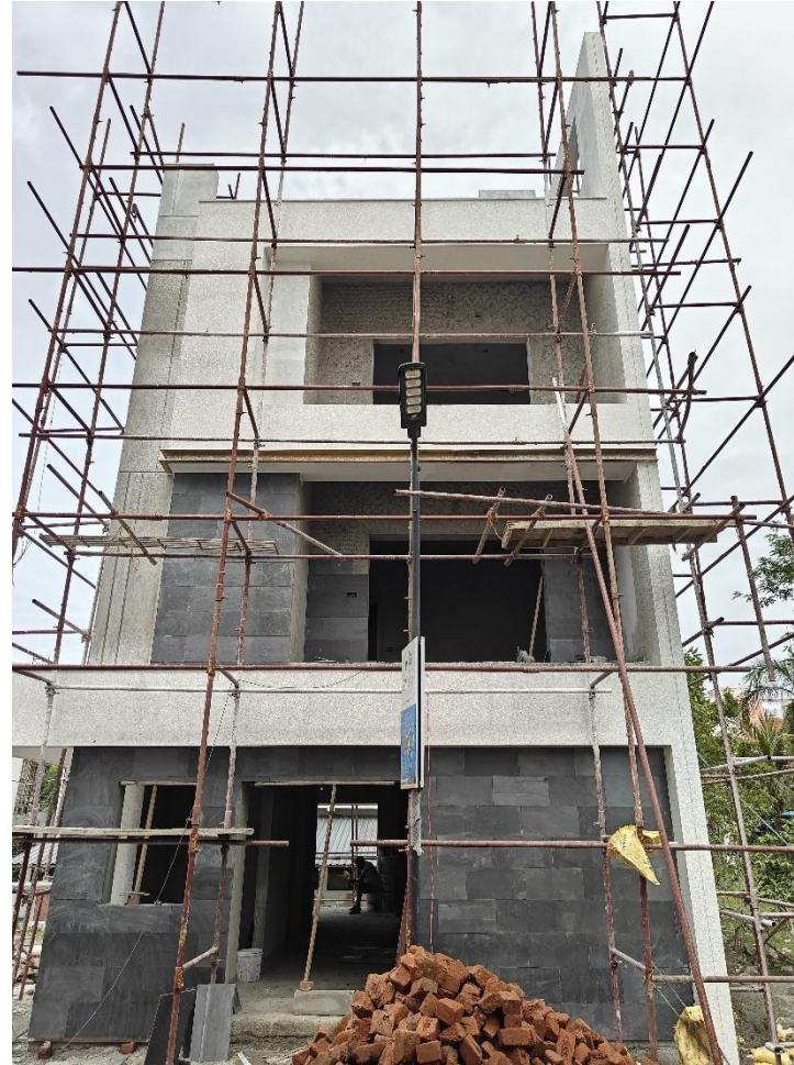
Villa No 3 – Front Elevation Slate tile laying work in progress
