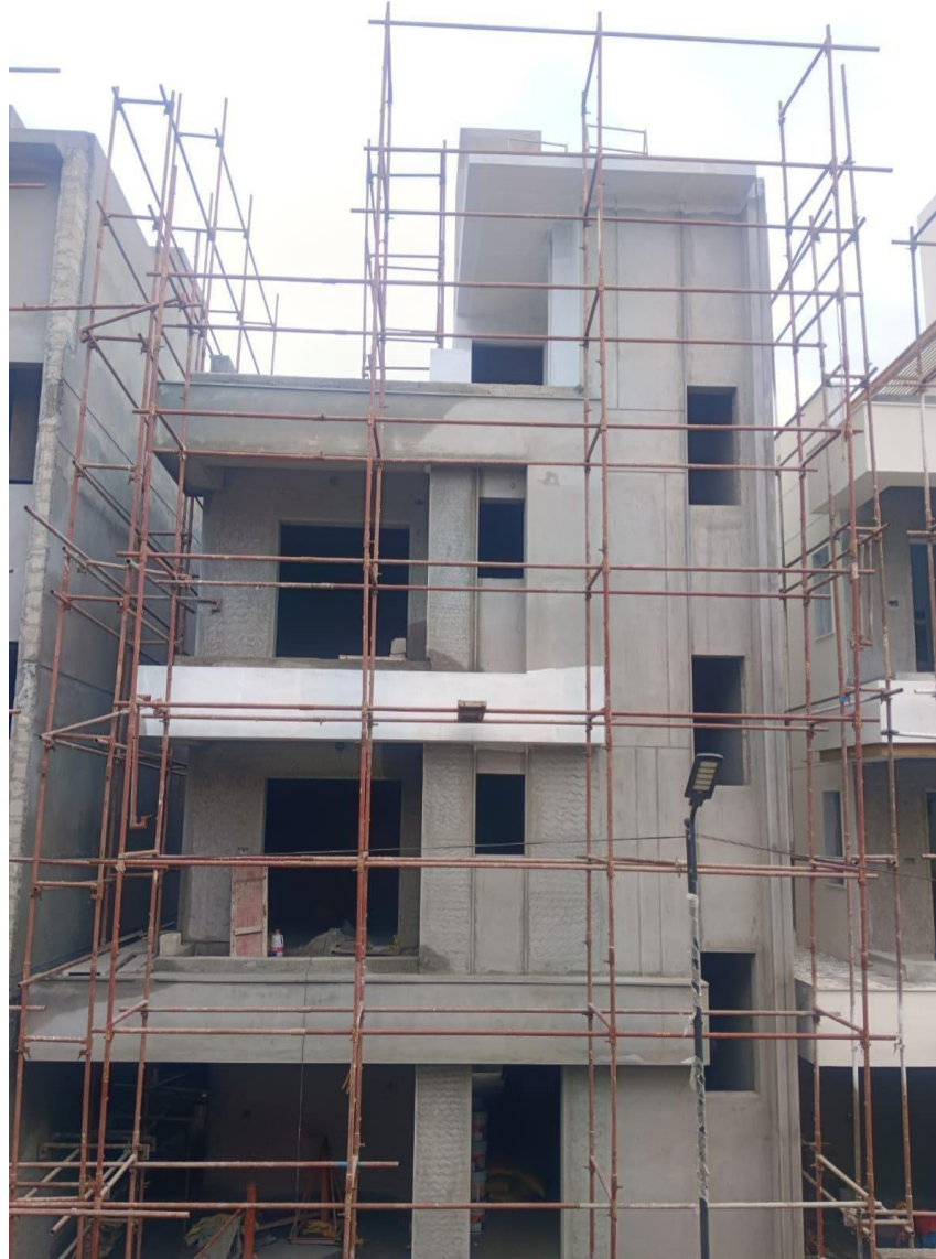
Villa No 8- Front elevation wall plastering work Completed
