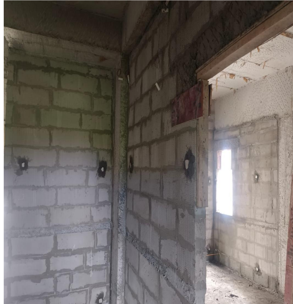
Villa No 15–FF Block Work Completed
