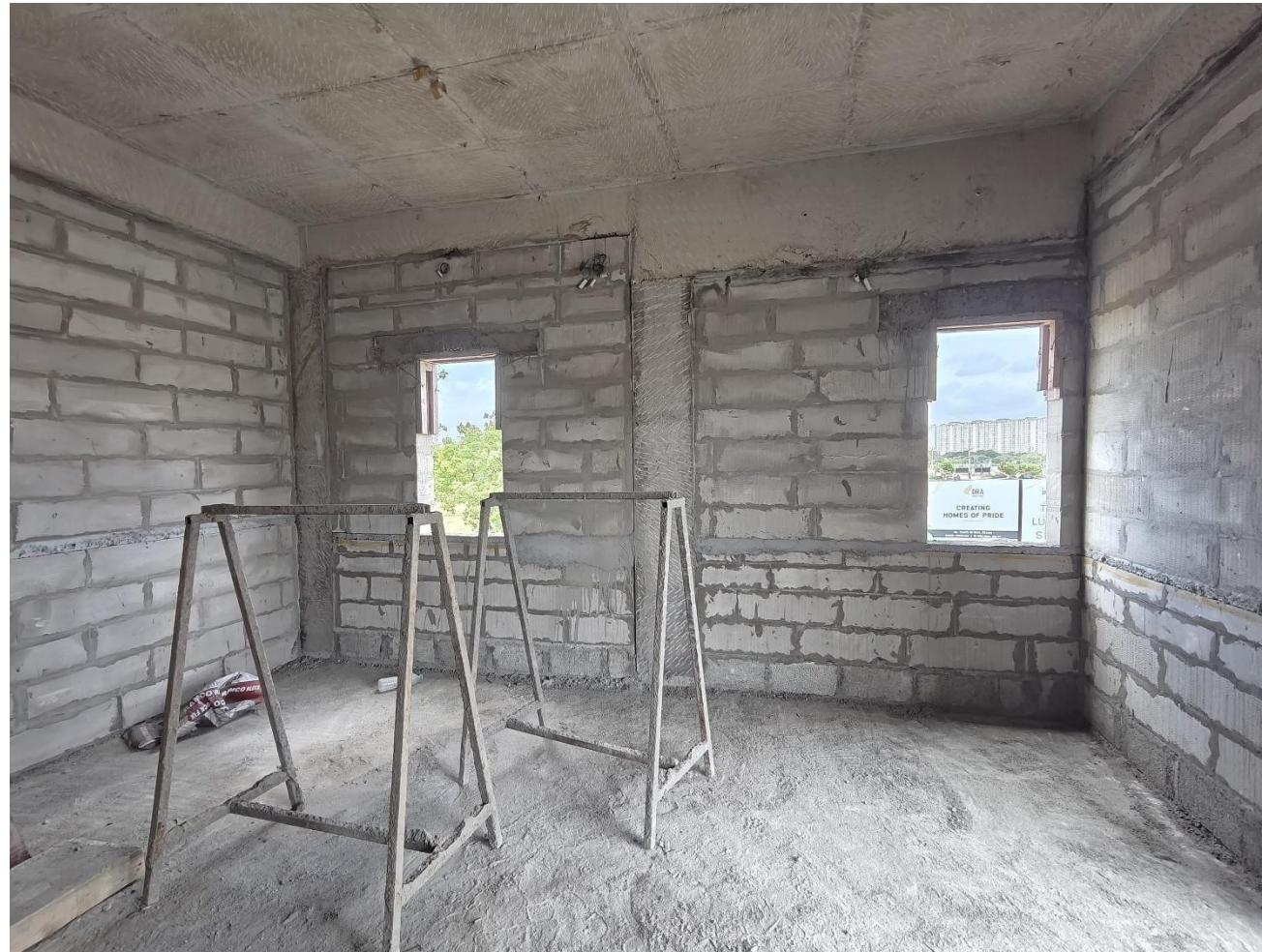
Villa No 17 – FF Bedroom blockwork in progress
