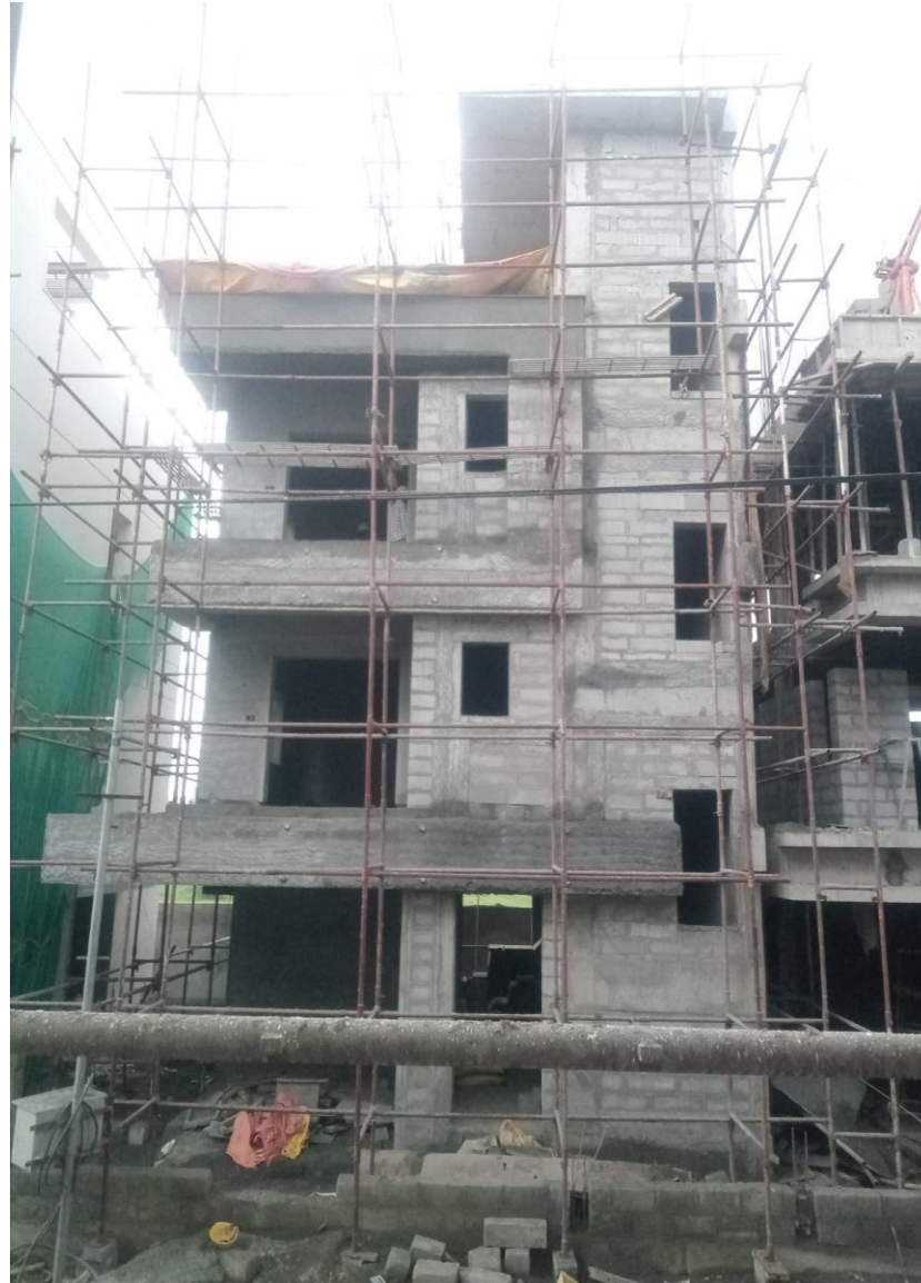
Villa No 13-Front elevation Plastering Preparation work in Progress
