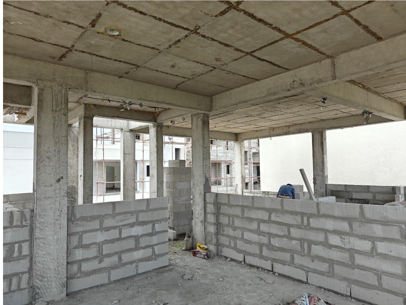
Villa No 17 – SF Bedroom blockwork in progress
