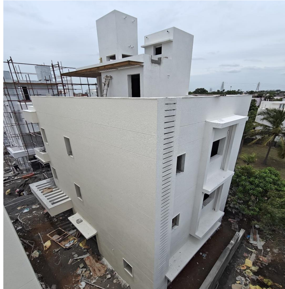
Villa No 4 – External wall pebble texture 1 st coat colour applying work in progress
