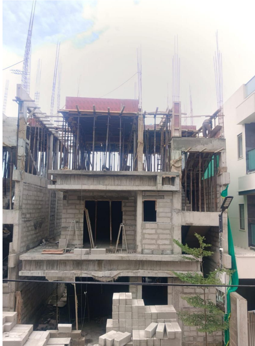
Villa No 15–SF Roof Slab Shuttering Work In Progress
