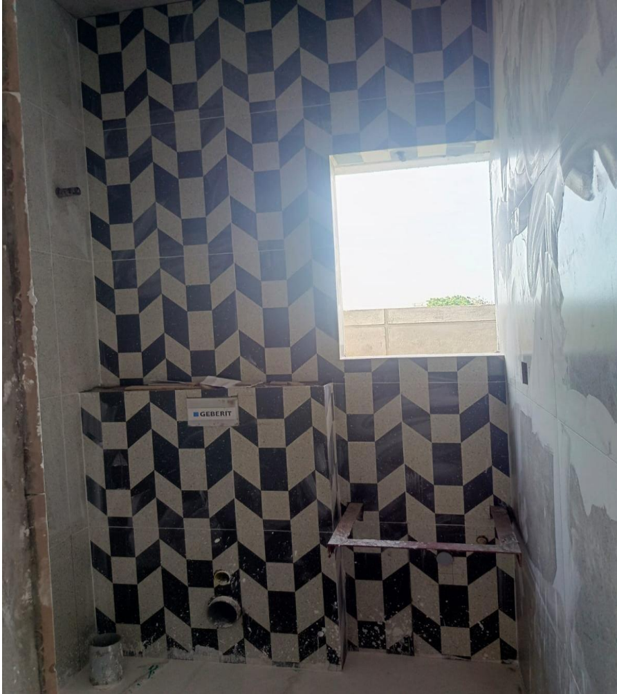
Villa No 12- GF Toilet Tiles Laying Work Completed
