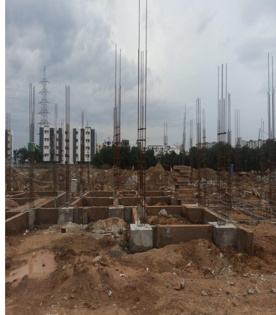
Phase 2 – villa no 50, 51 plinth beam concrete pouring Completed
