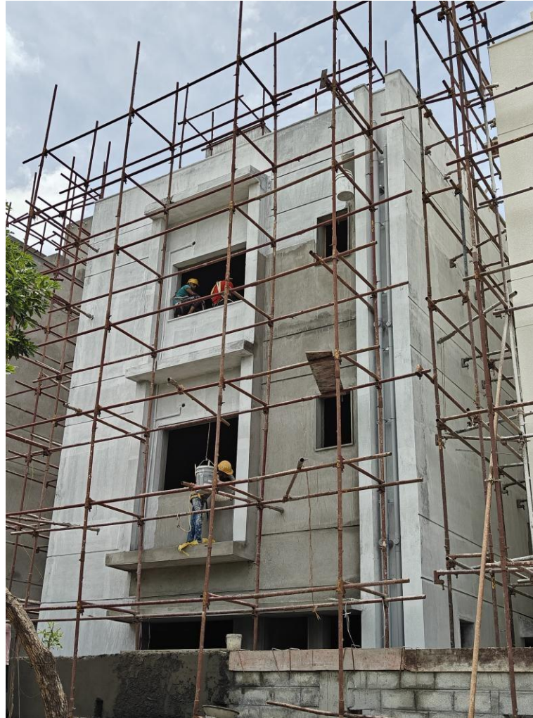
VillaNo 10- Backside external primer coat applying work in progress
