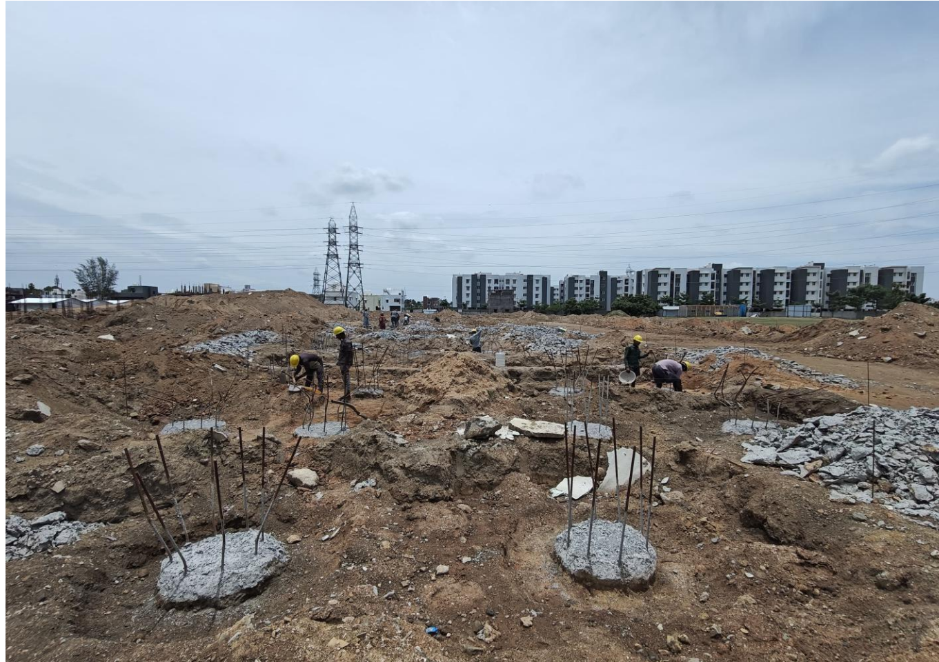
Phase 2 – villa no 67 , 68 pile cap concrete chipping work in progress
