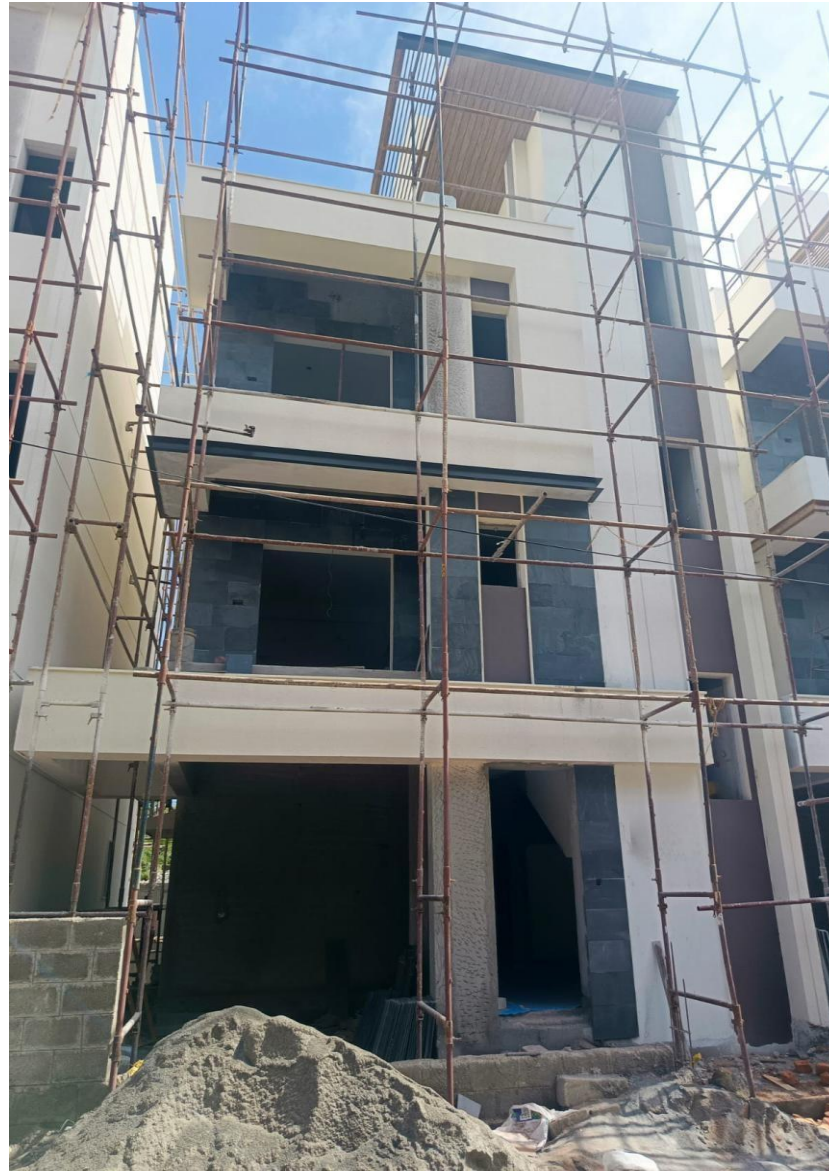
Villa No 9 –Front Elevation Slate Tiles Laying work in progress
