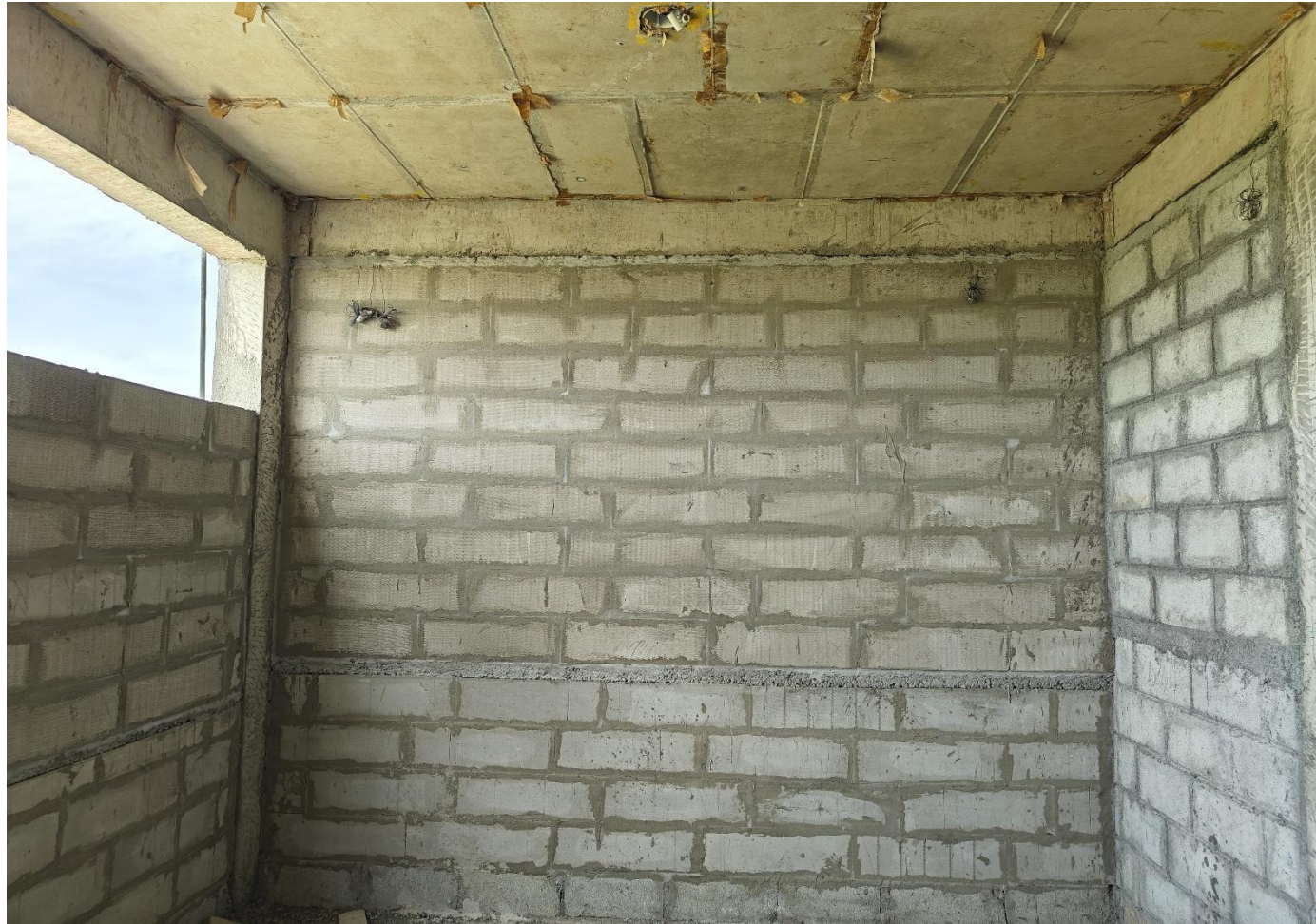
Villa No 14– FF Bedroom blockwork in progress
