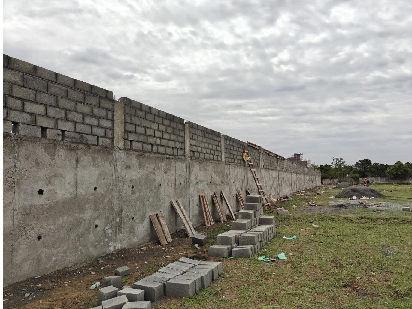
Phase 2 - Southside compound wall blockwork in progress
