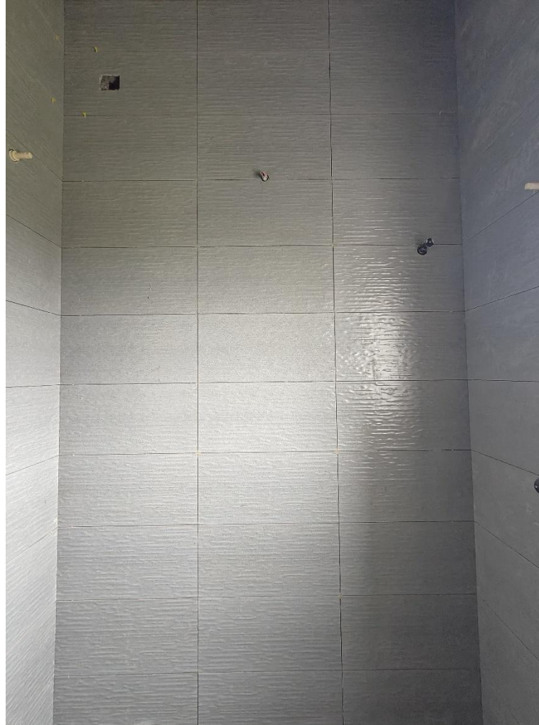
Villa No 6- FF Bedroom toilet wall tile laying work in progress
