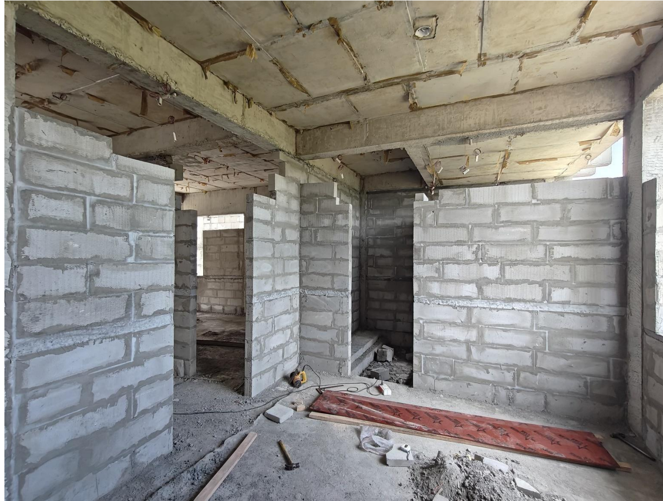
Villa No 15– First Floor blockwork in progress
