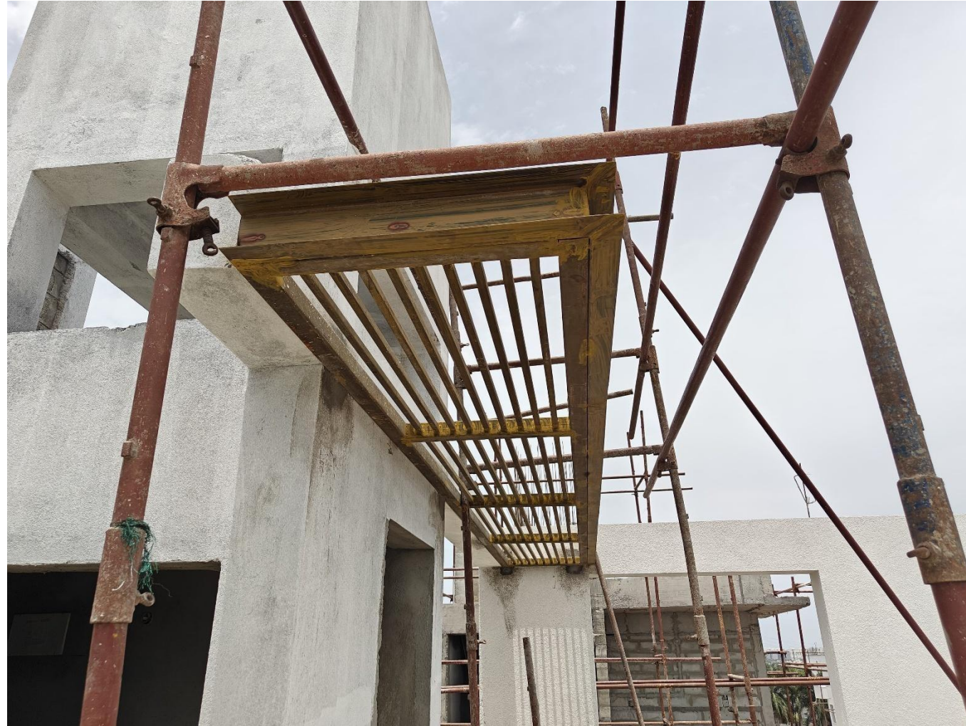
Villa No 12 – Terrace area M.S Percola fixing work in progress
