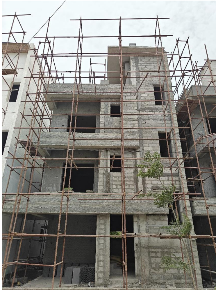
Villa No 7- Front Elevation wall plastering preparation work in progress
