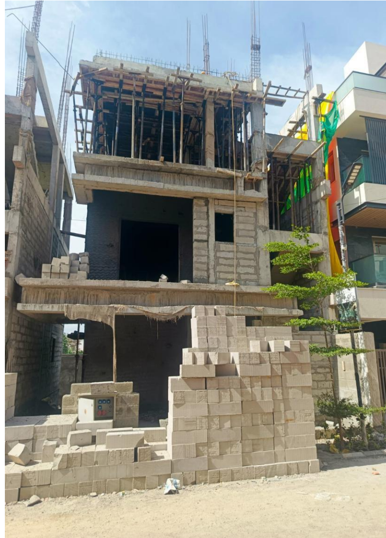
Villa No 15 –SF Roof Slab Concrete Completed
