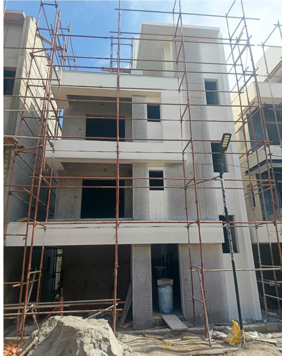
Villa No 8-Front elevation primer applying work in Completed
