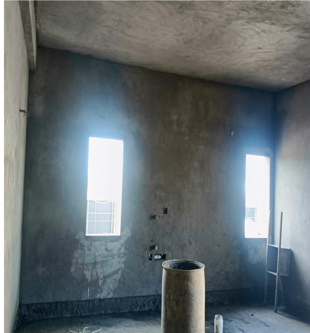
Villa No-17 FF Plastering Work In Progress
