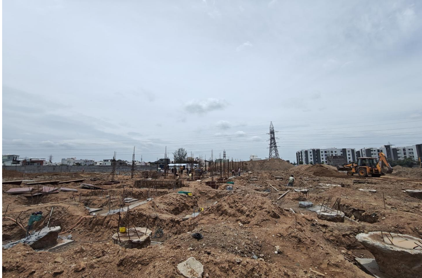
Phase 2 – villa no 54 pile cap concrete chipping work in progress
