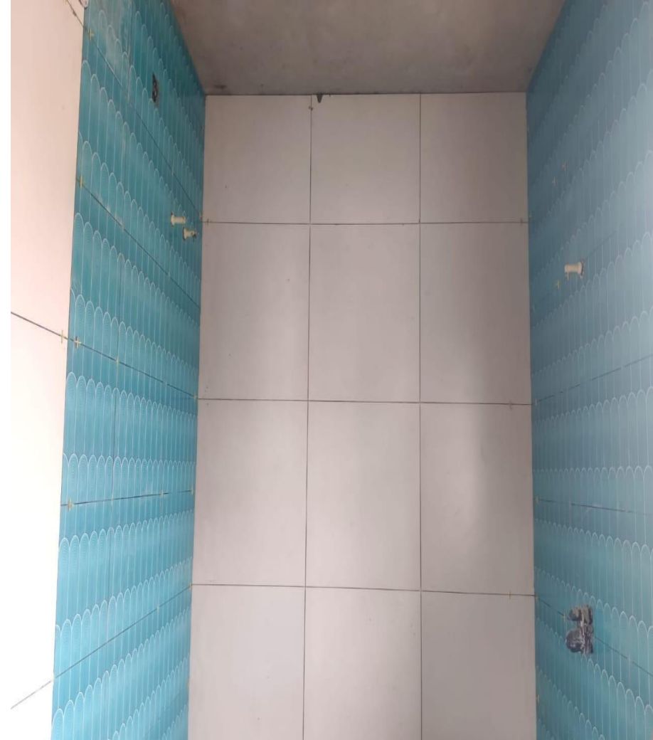
Villa No 3- FF Toilet wall Tile Laying work in progress
