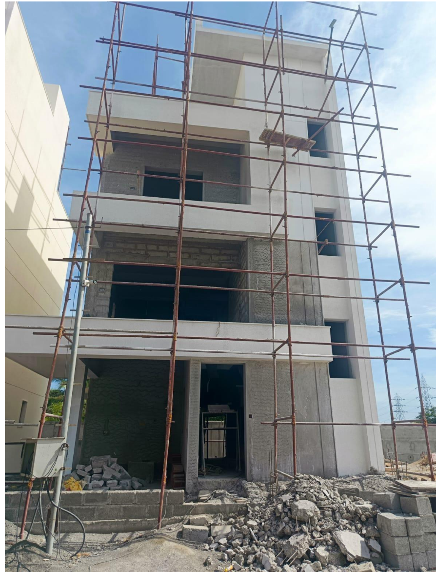
Villa No 11-Front elevation Arch Concrete Putty Applying Work Progress
