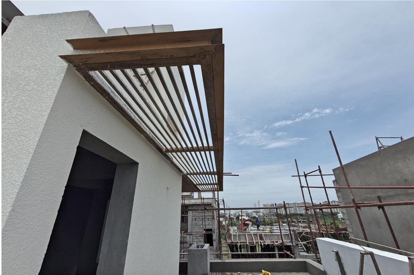
Villa No 9 – Terrace area MS Percola fixing work in progress
