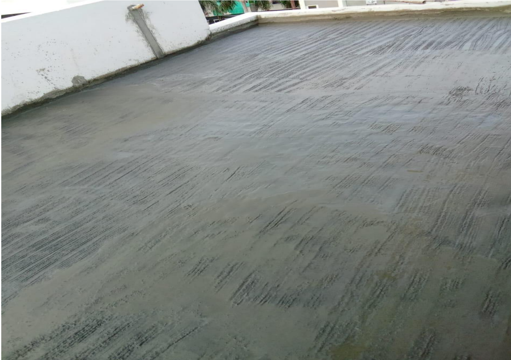
Villa No 5 – Treece area weathering course Completed
