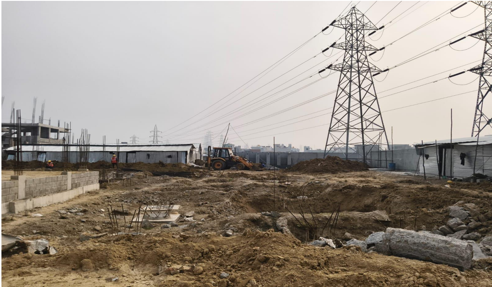
Villa No 82 – Pile Chipping work In Progress
