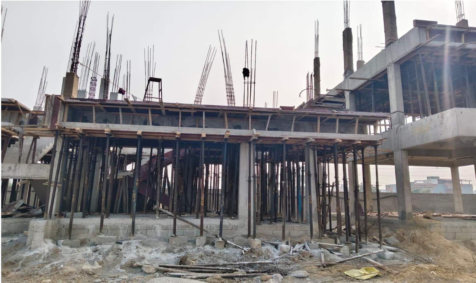
Villa No 28 –FF Column Reinforcement Work Completed
