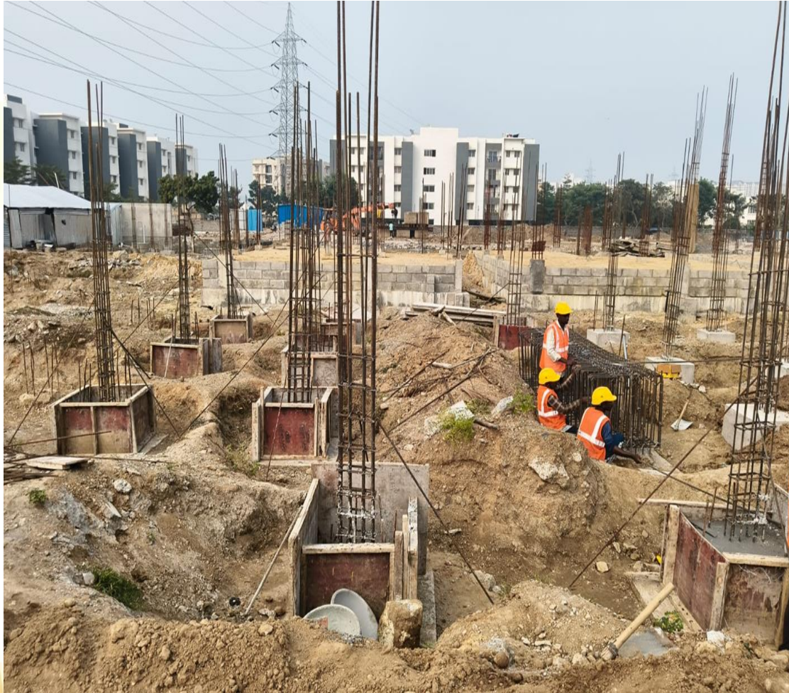
Villa - 63 –Pile Cap Shuttering Work InProgress.
