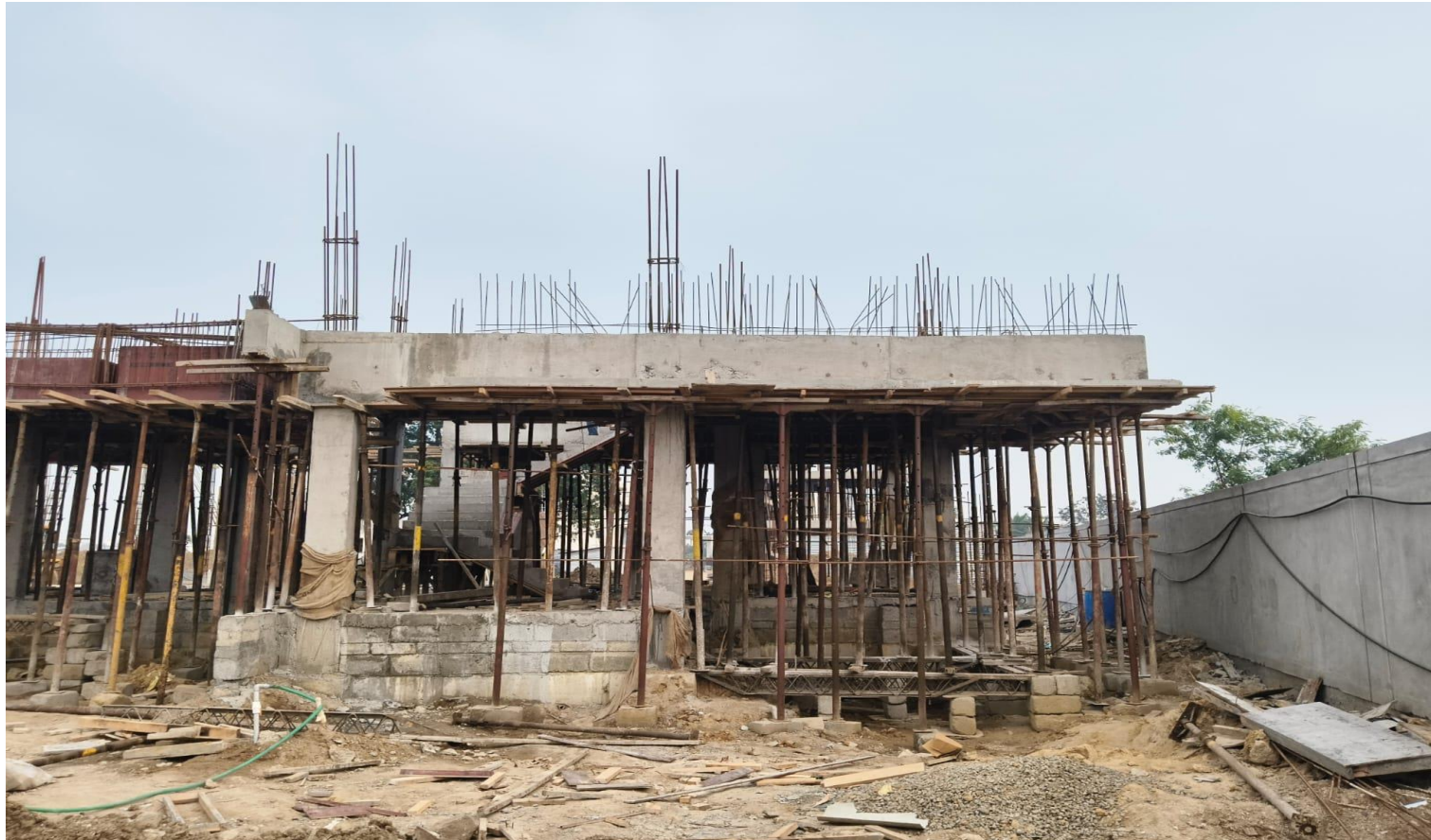
Villa No 38–GF Roof Slab Concrete Completed
