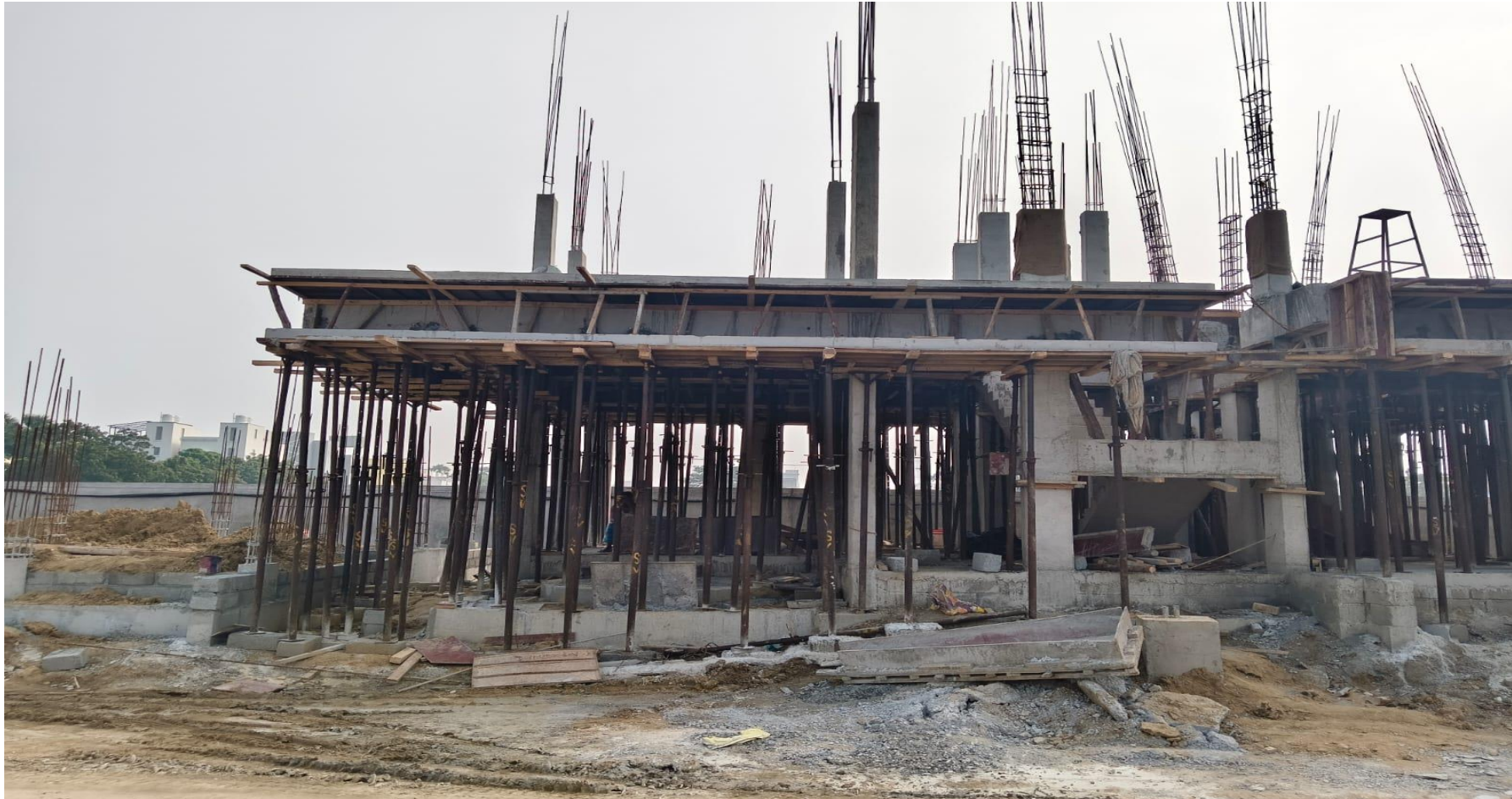
Villa No 27–FF Column Concrete work Completed
