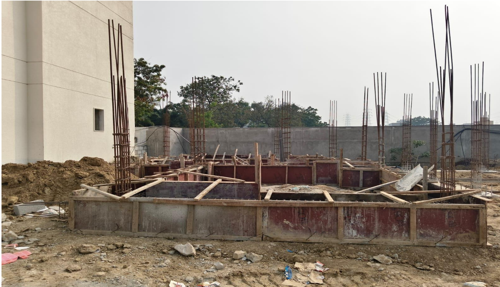
Villa No 22 –Plinth Beam Shuttering work Completed
