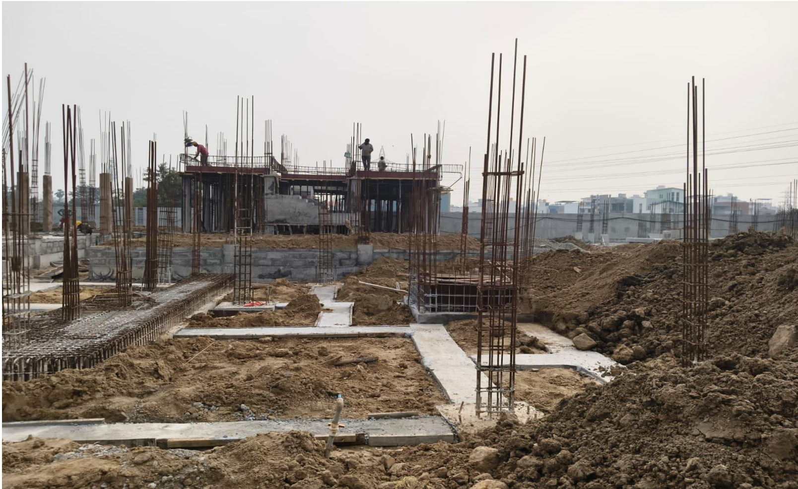
Villa No 35 –Plinth Beam PCC Completed
