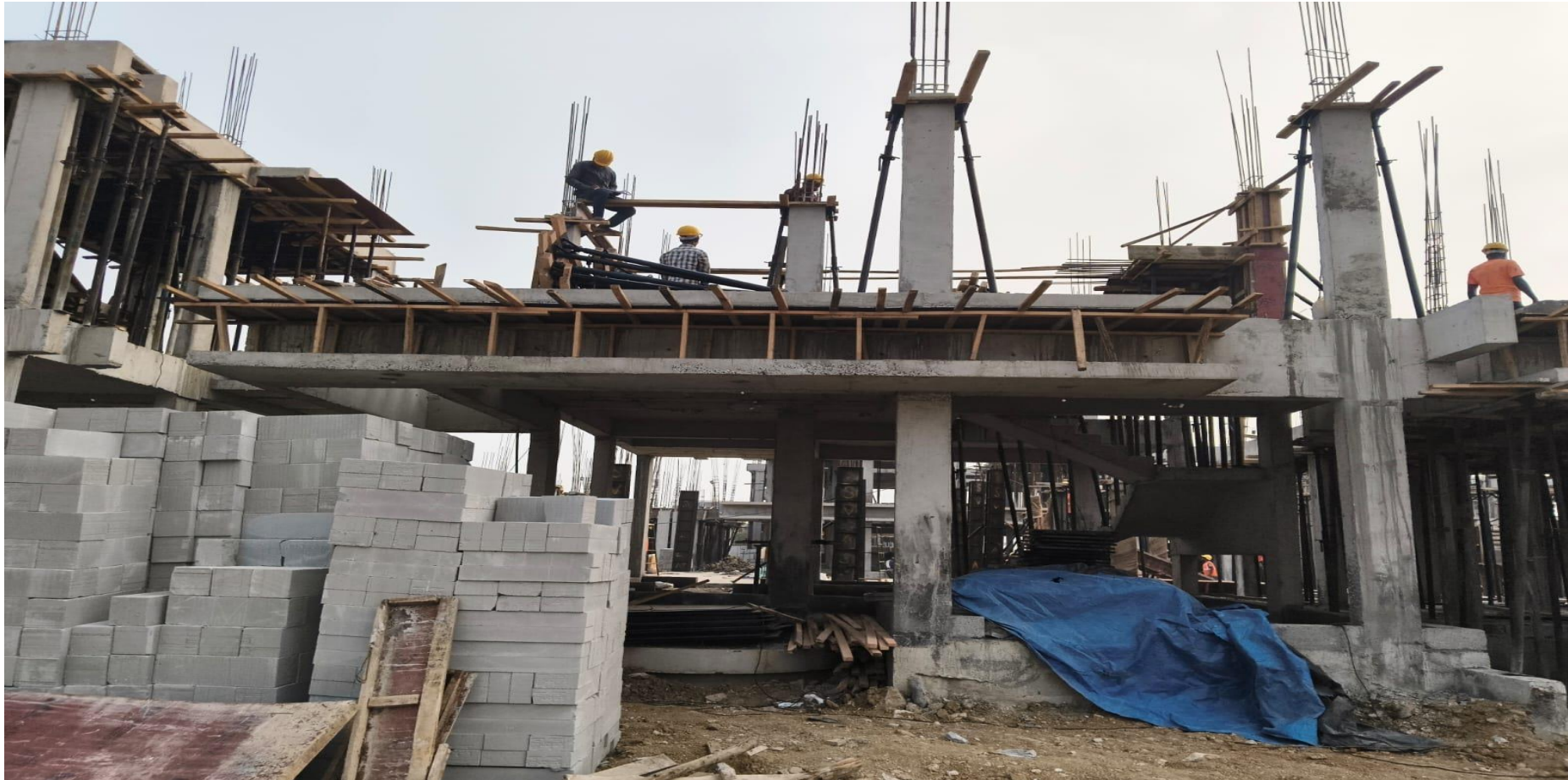
Villa No 74 –FF Roof Slab Shuttering Work In Progress
