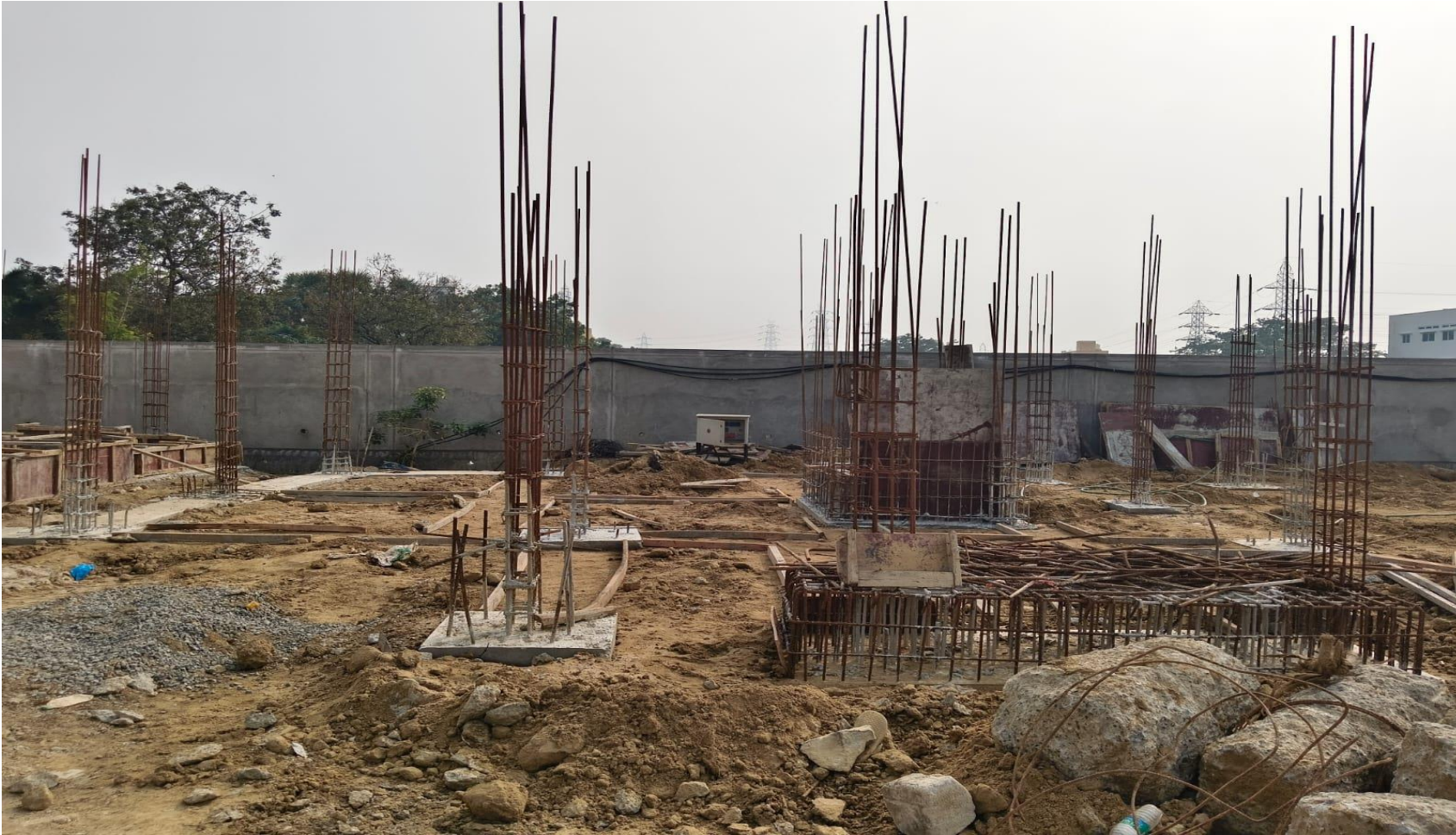
Villa No 23 –Plinth Beam PCC work In Progress
