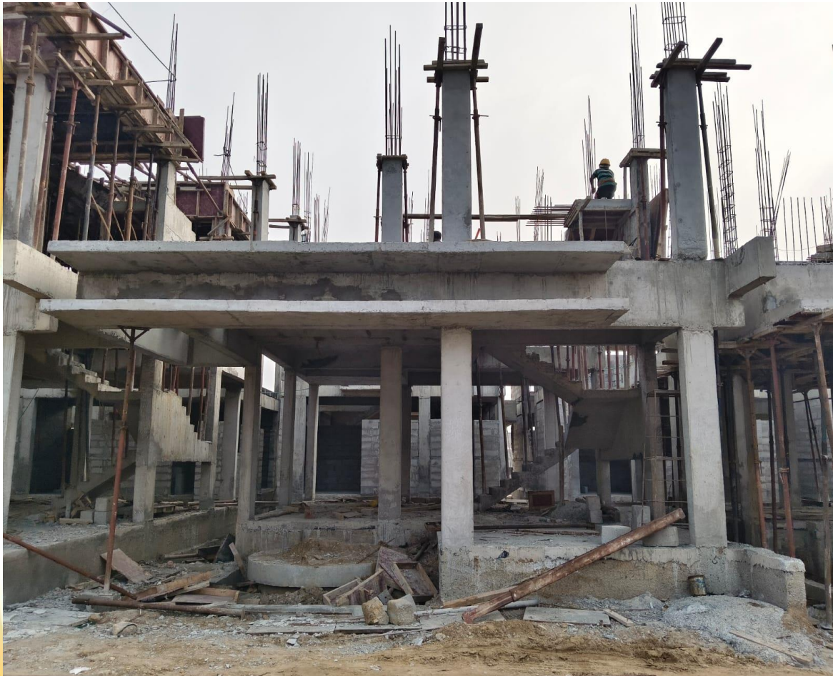
Villa - 59 - 1 st Floor Roof Slab Shuttering WIP.
