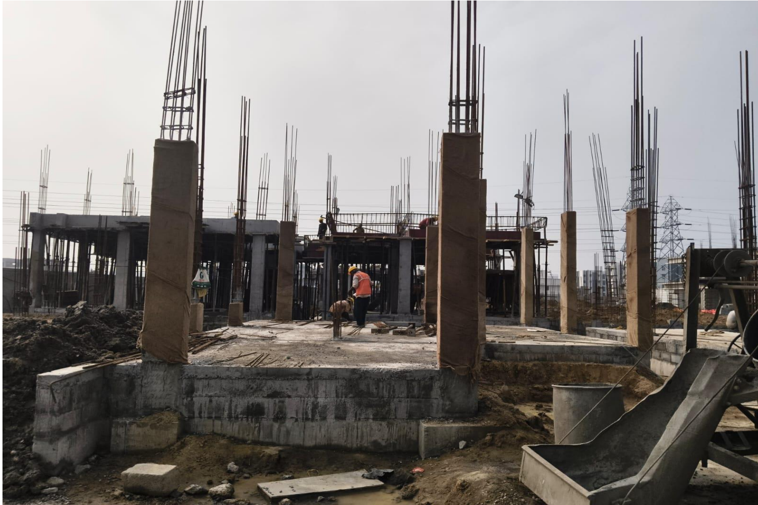
Villa No 31-GF column concrete completed
