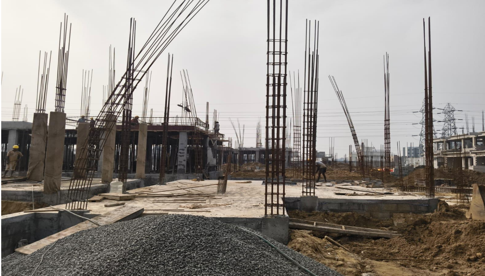
Villa No 32 – GF column reinforcement progress
