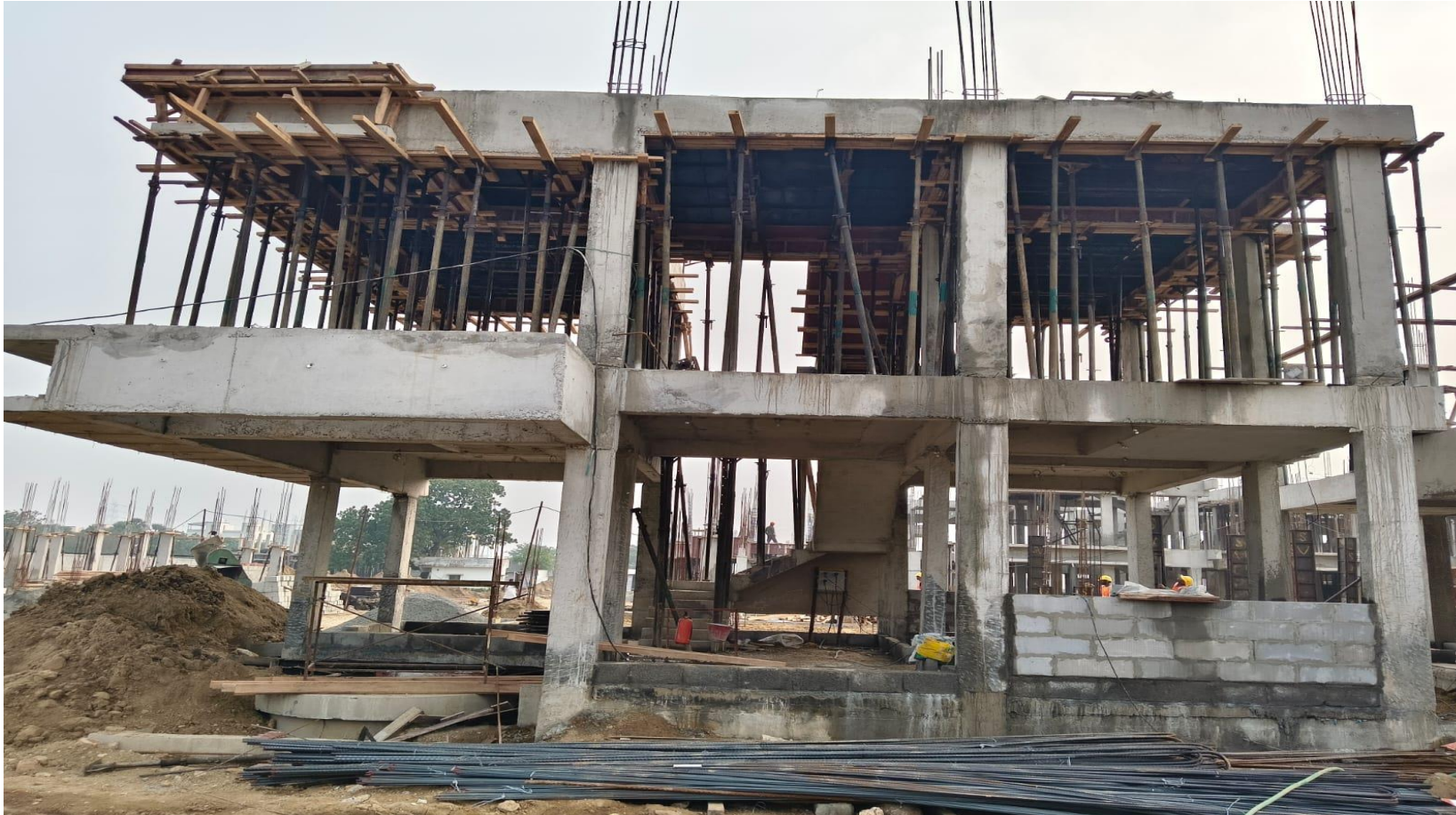
Villa No 73 –FF Roof Slab Concrete Completed
