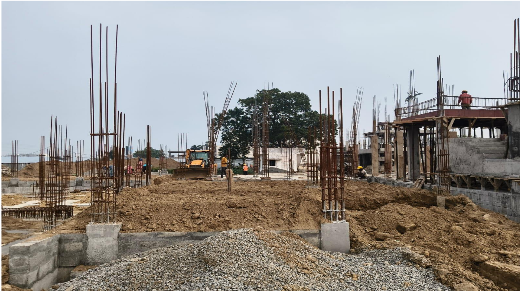
Villa No 36–Basement Back Filling Work In Progress
