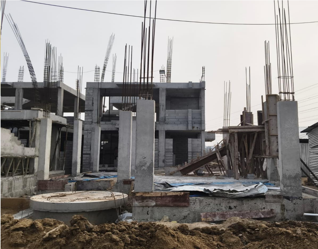
Villa - 61 -G Floor Column Completed.
