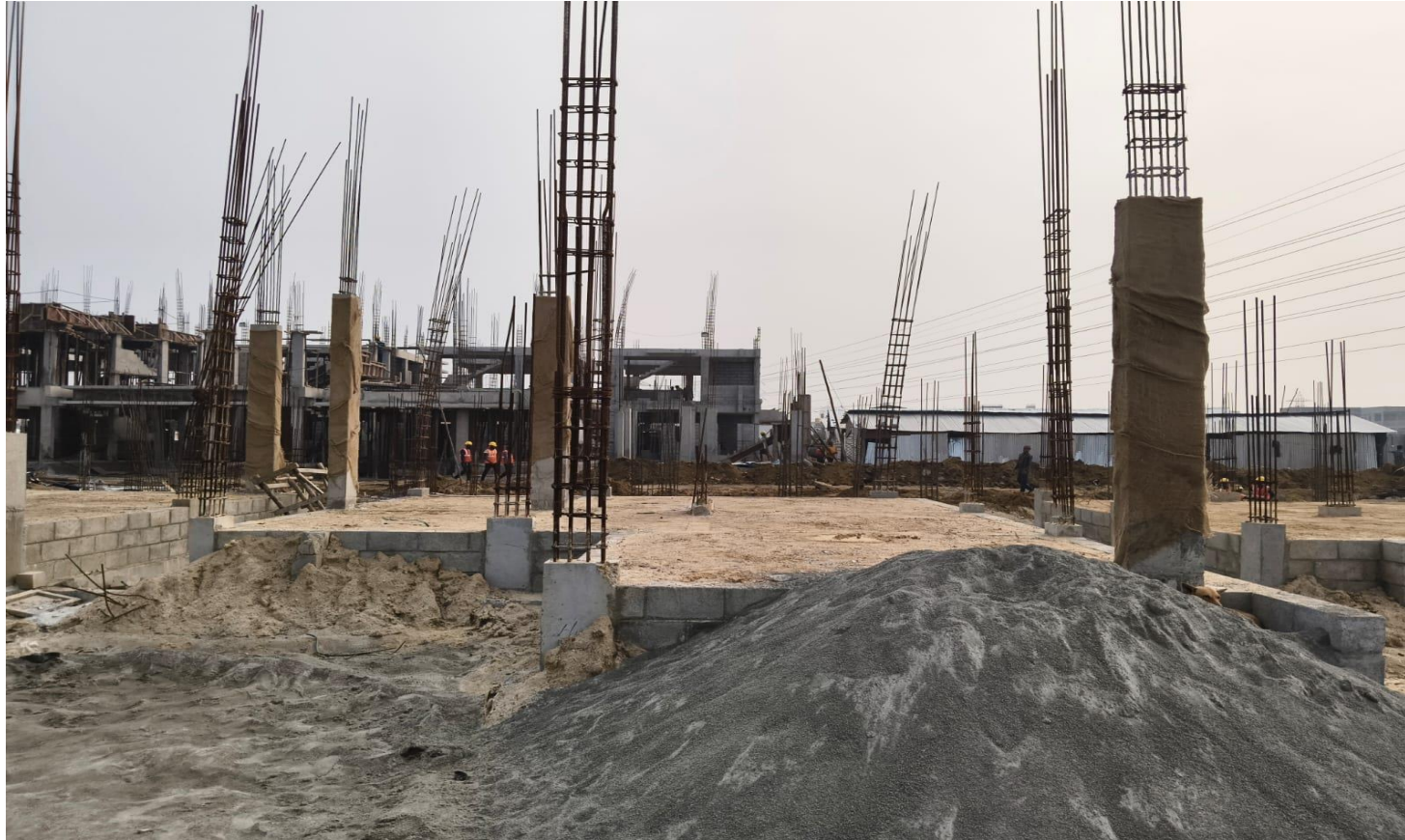
Villa No 79 –GF column concrete completed
