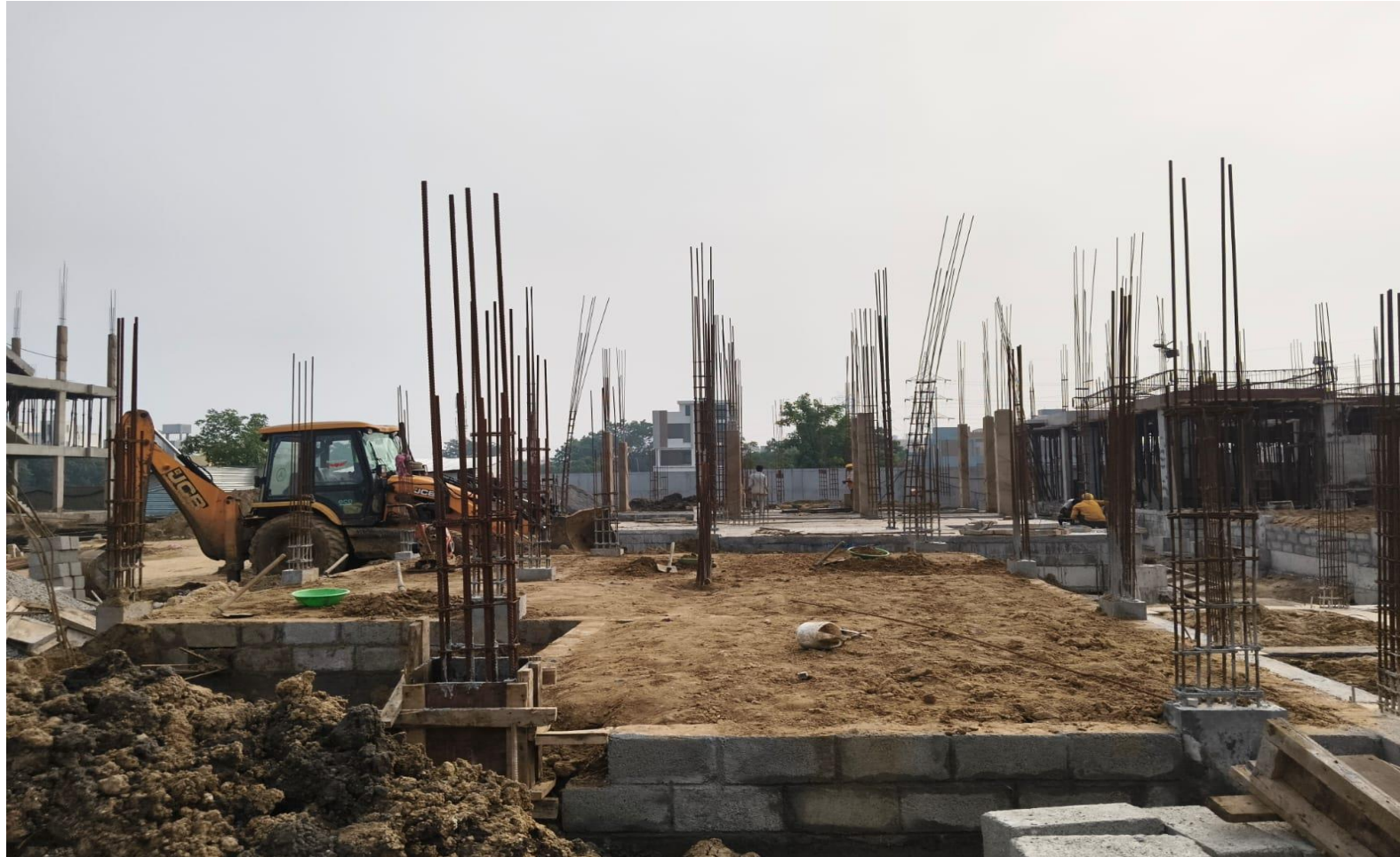
Villa No 33 –Basement Back Filling work Completed
