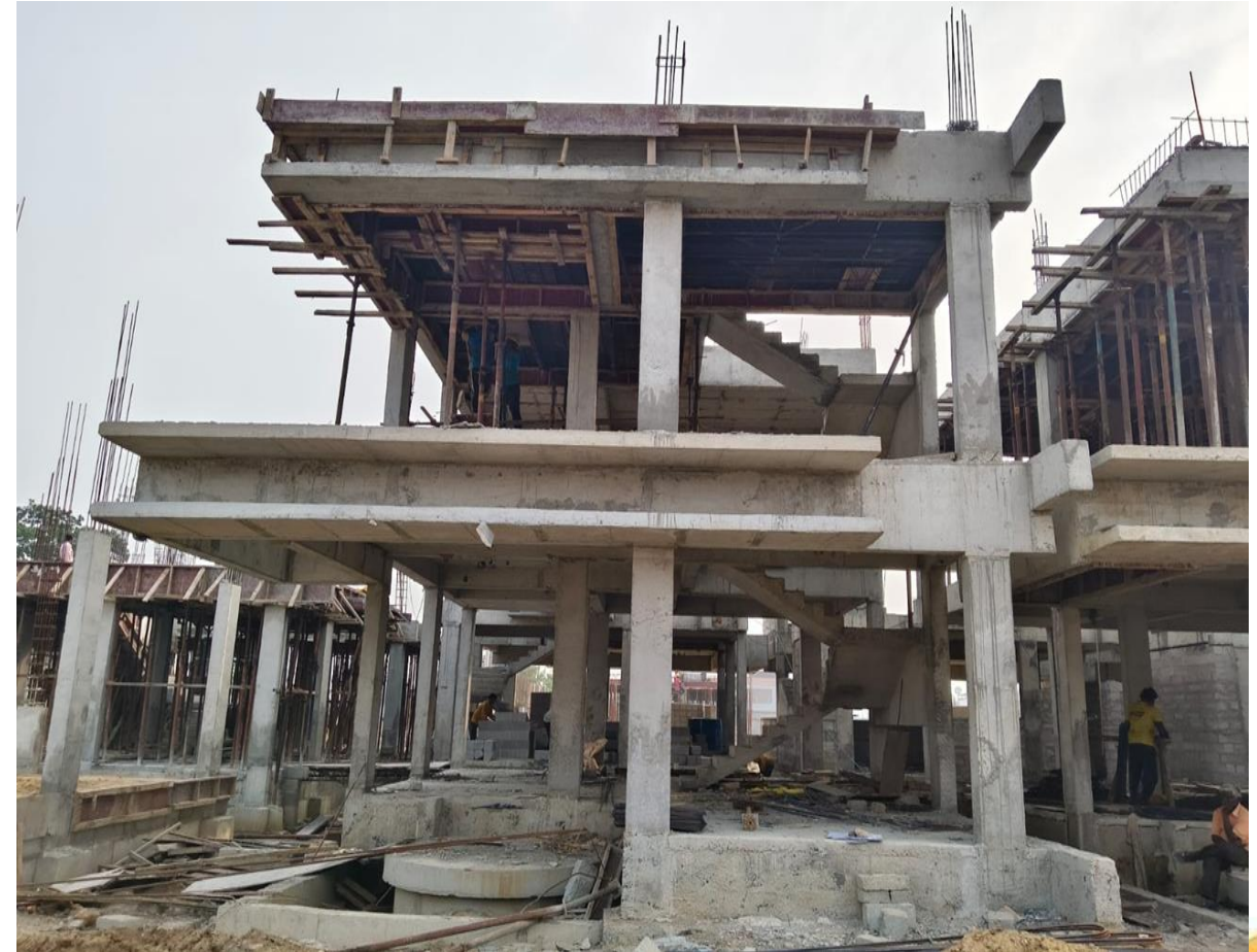
Villa - 56 - 1 st Floor Roof Slab Completed.
