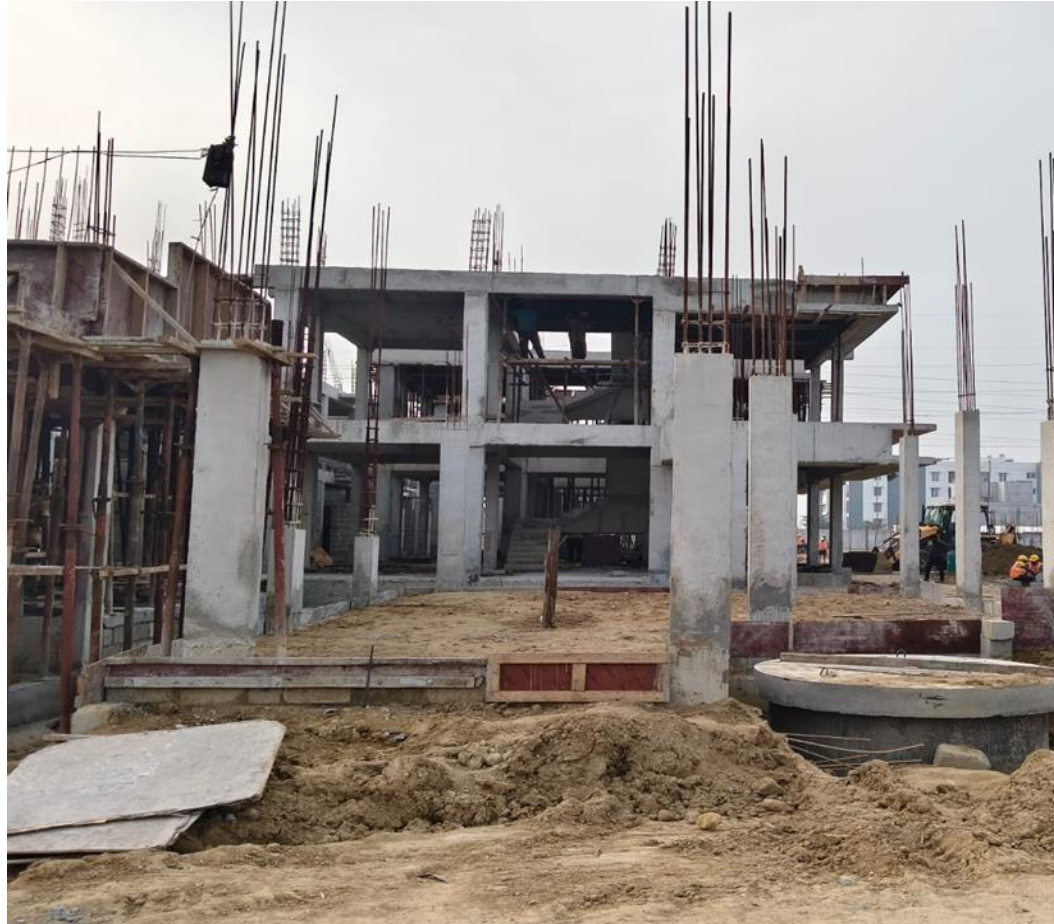
Villa - 55 -GF Column Concrete Completed.
