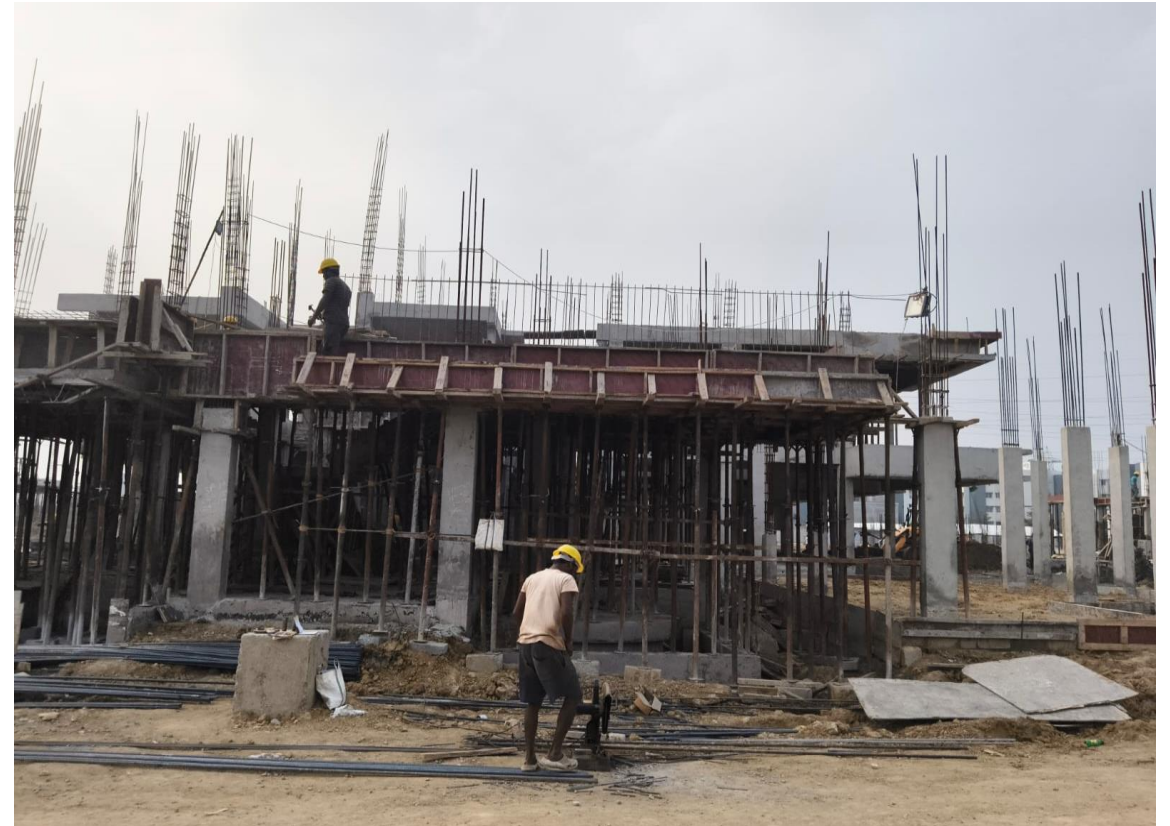
Villa - 54 - 1 st Floor Column RCC Work In Progress
