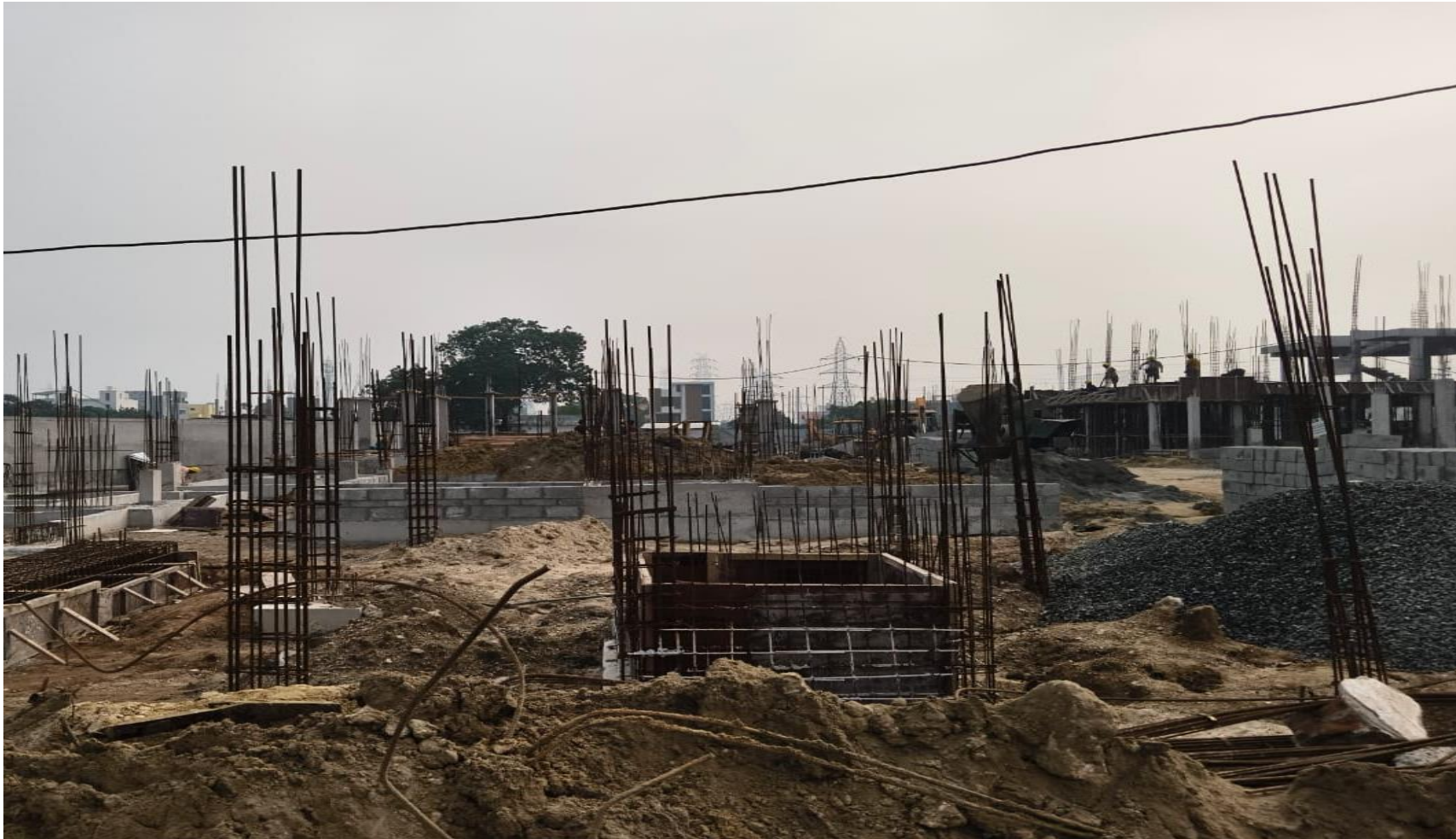
Villa No 105 – Pile Cap Concrete Work Completed
