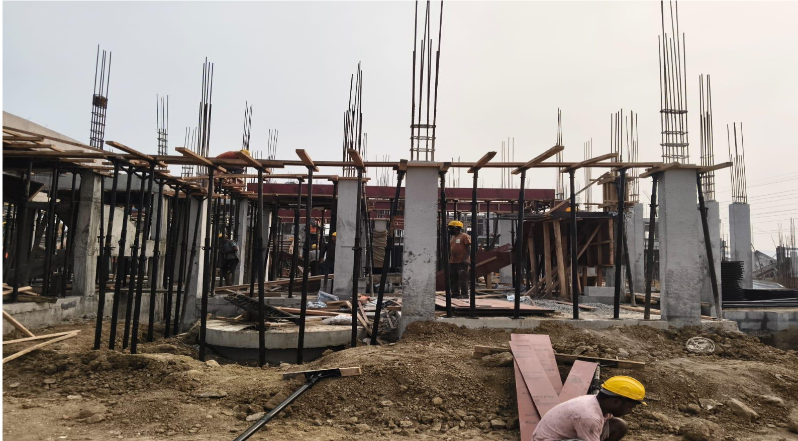
Villa No 76 –GF Roof Slab Shuttering Work In Progress
