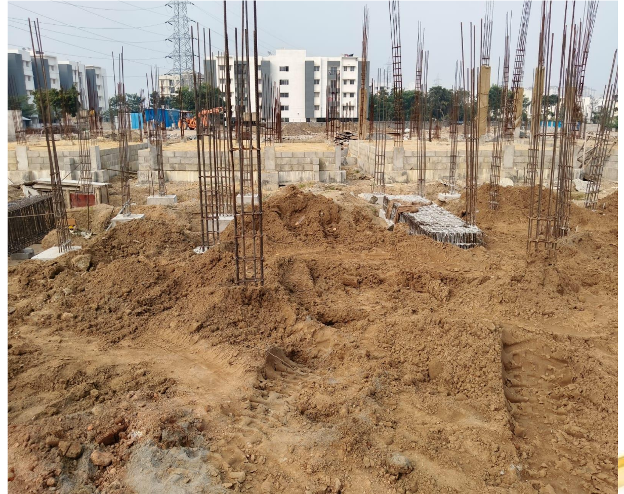
Villa - 64 – Pile Cap Concrete Completed.
