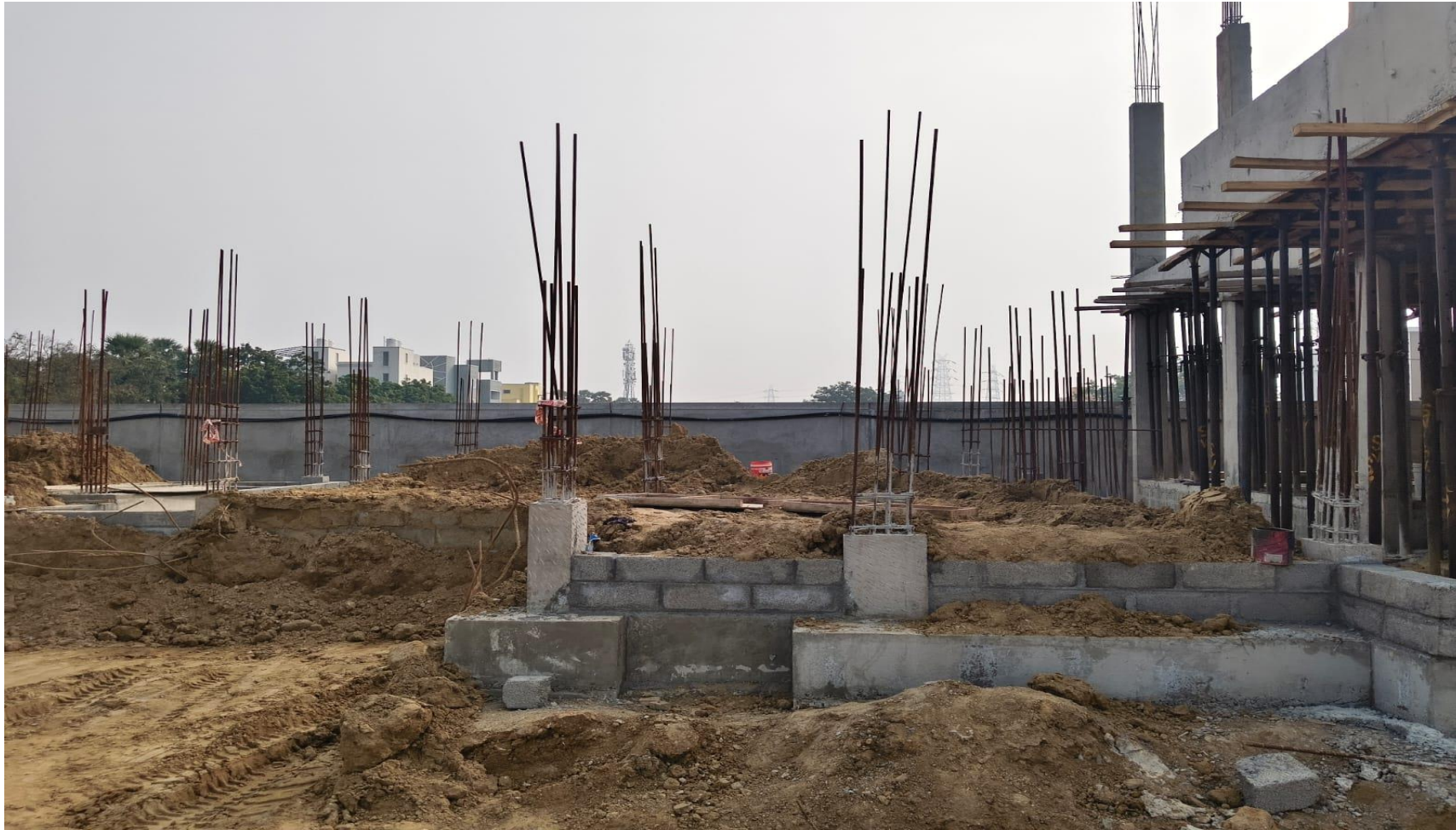
Villa No 26- Basement Back Filling work Completed
