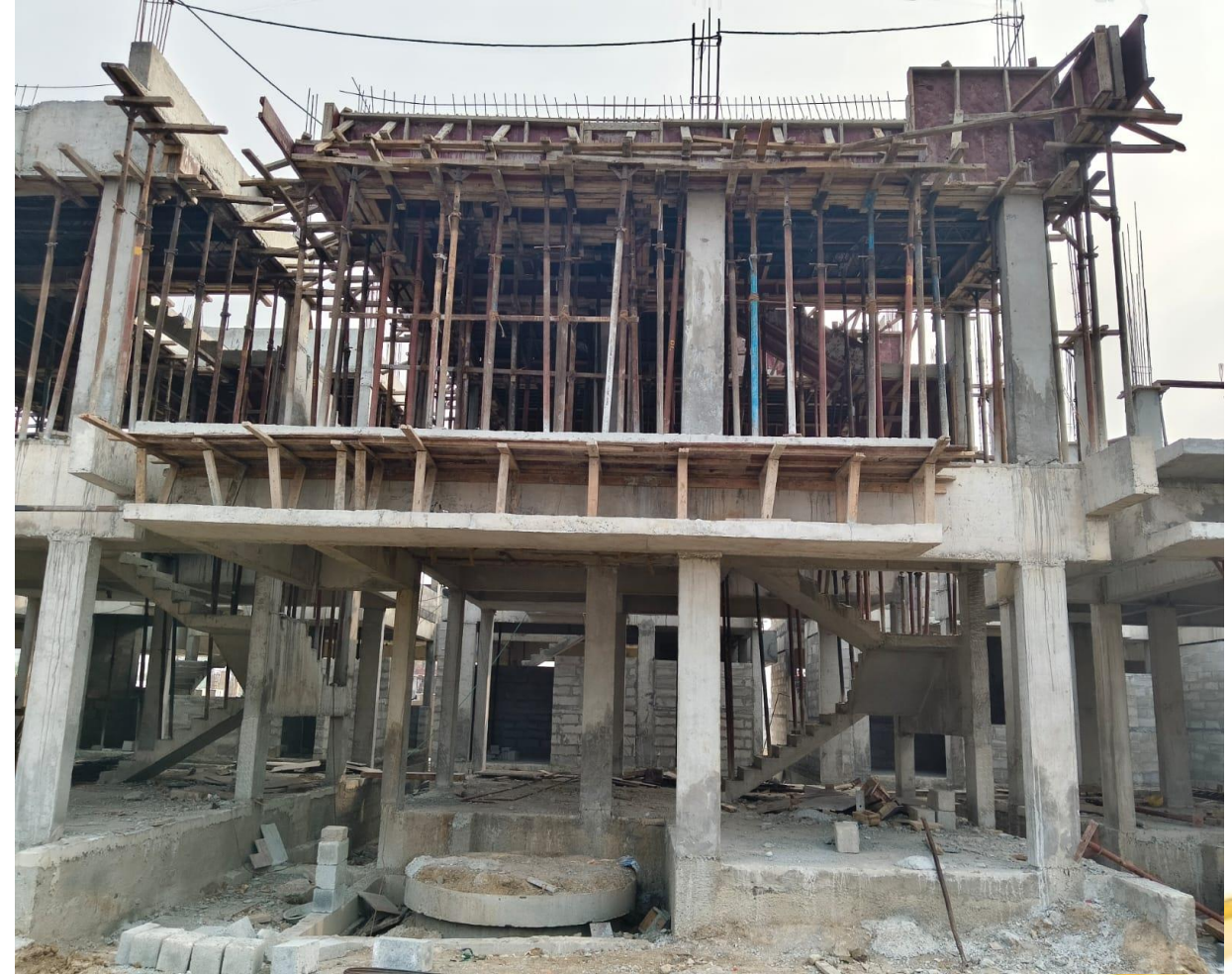
Villa - 58 - 1 st Floor Roof Slab Completed.
