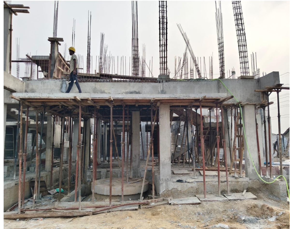
Villa - 60 - 1 st Floor Column RCC WIP.
