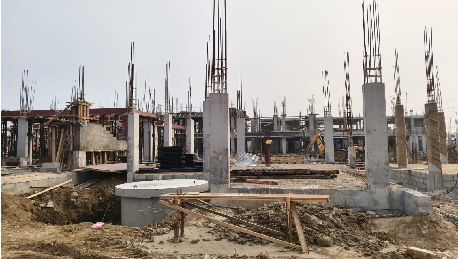
Villa No 77 –GF column concrete completed
