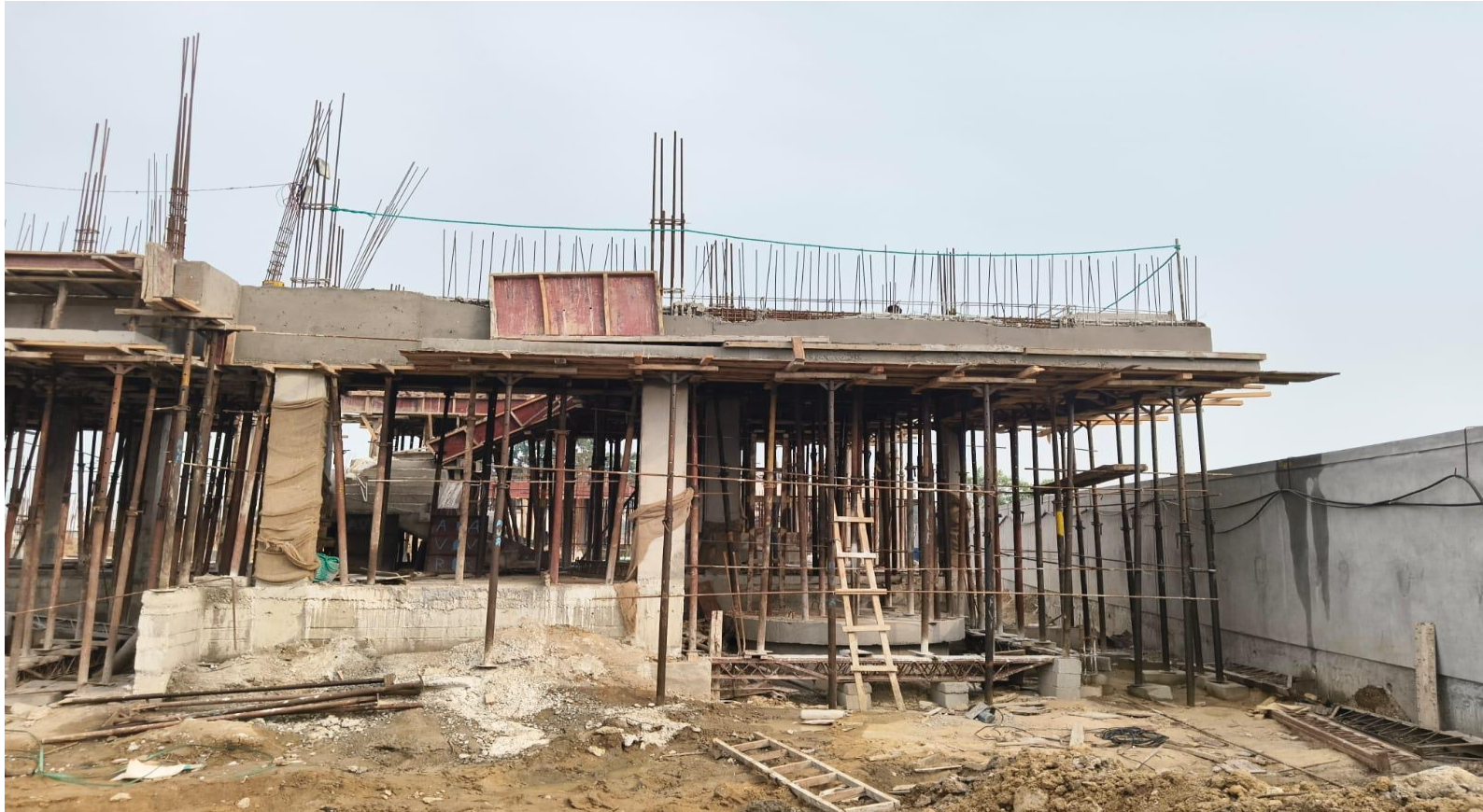
Villa No 45 –FF Column Reinforcement Work In Progress
