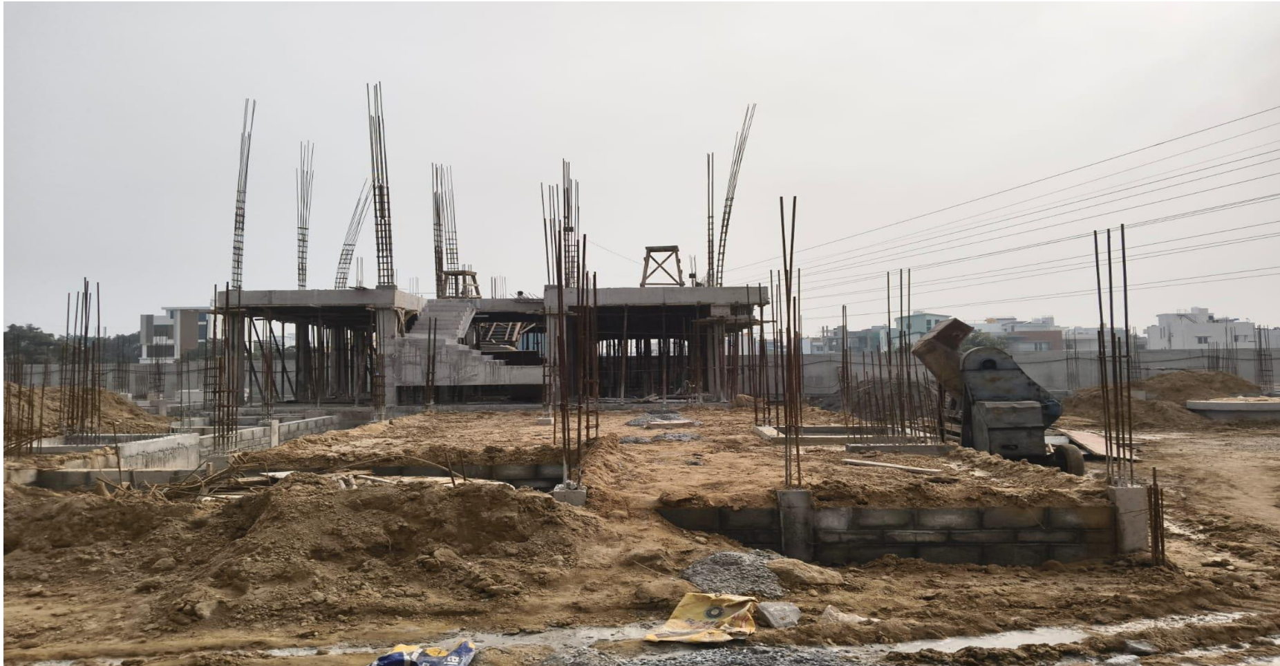
Villa No 43 –Basement Back Filling Work In Progress
