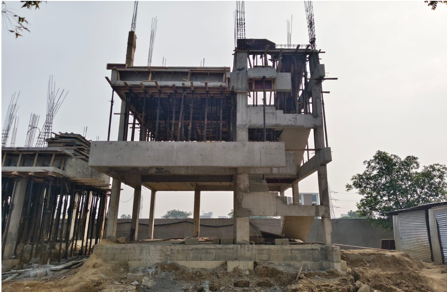
Villa No-29 SF Column Concrete Completed
