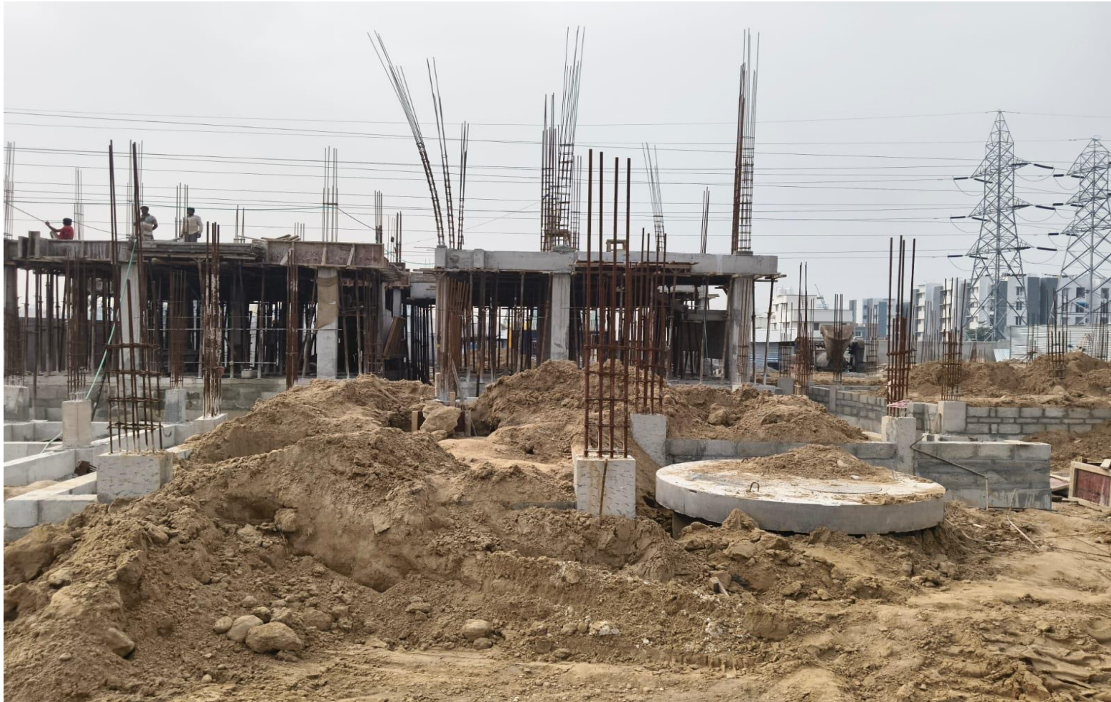
Villa No 40–Basement Back Filling Work In Progress
