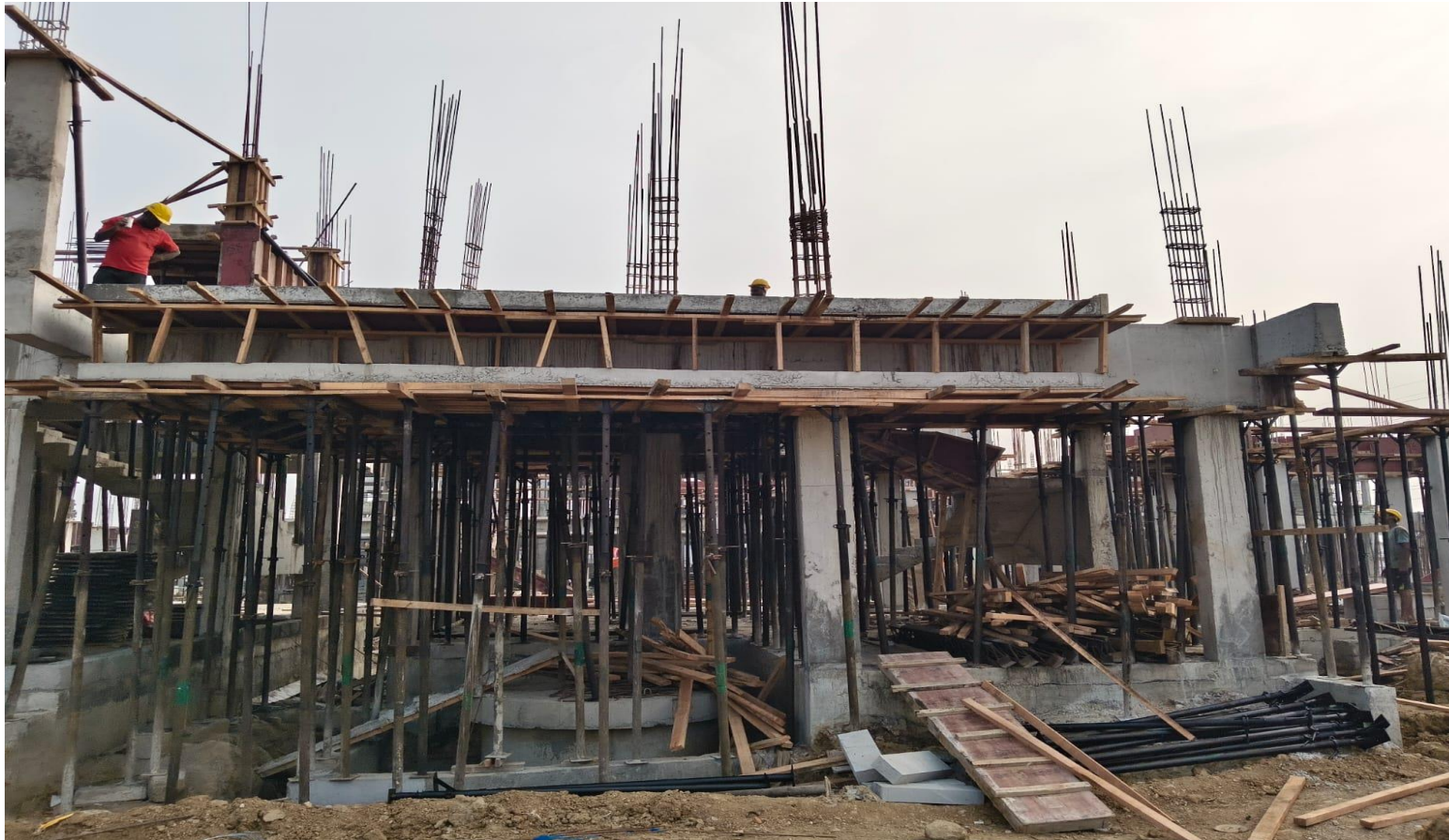
Villa No 75 –FF Column Reinforcement Work In Progress
