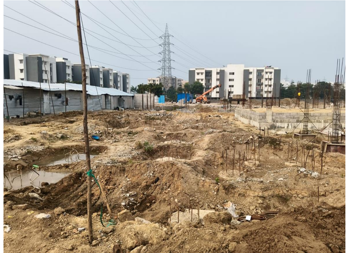
Villa - 62 - Pile Chipping Completed.
