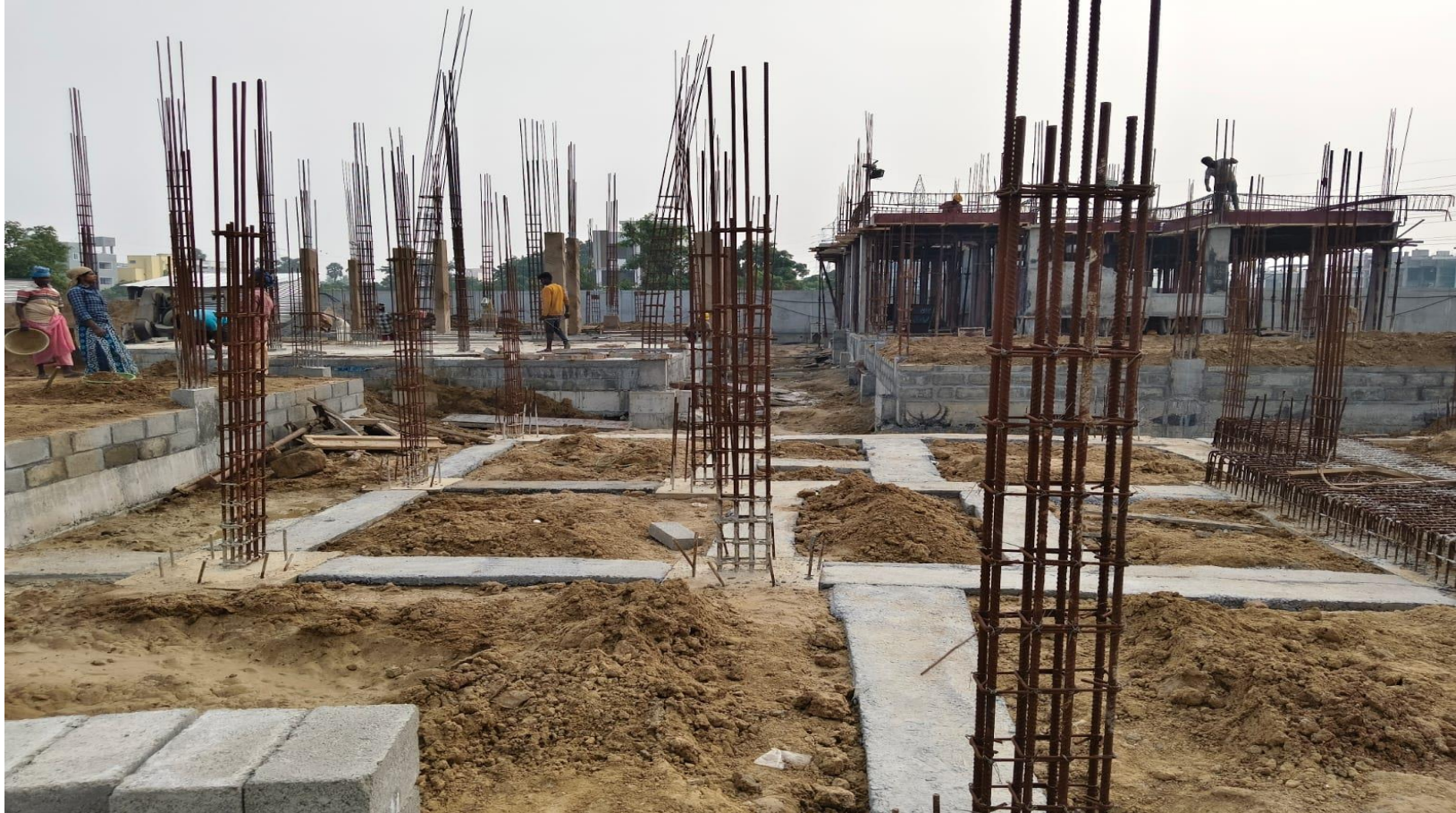
Villa No 34 – Plinth Beam PCC Completed
