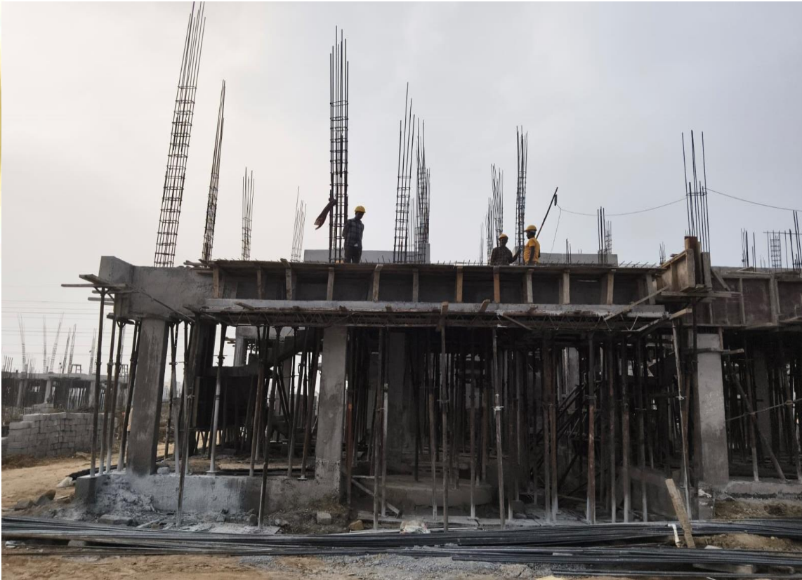
Villa - 53 - 1 st Floor Column RCC Work In Progress
