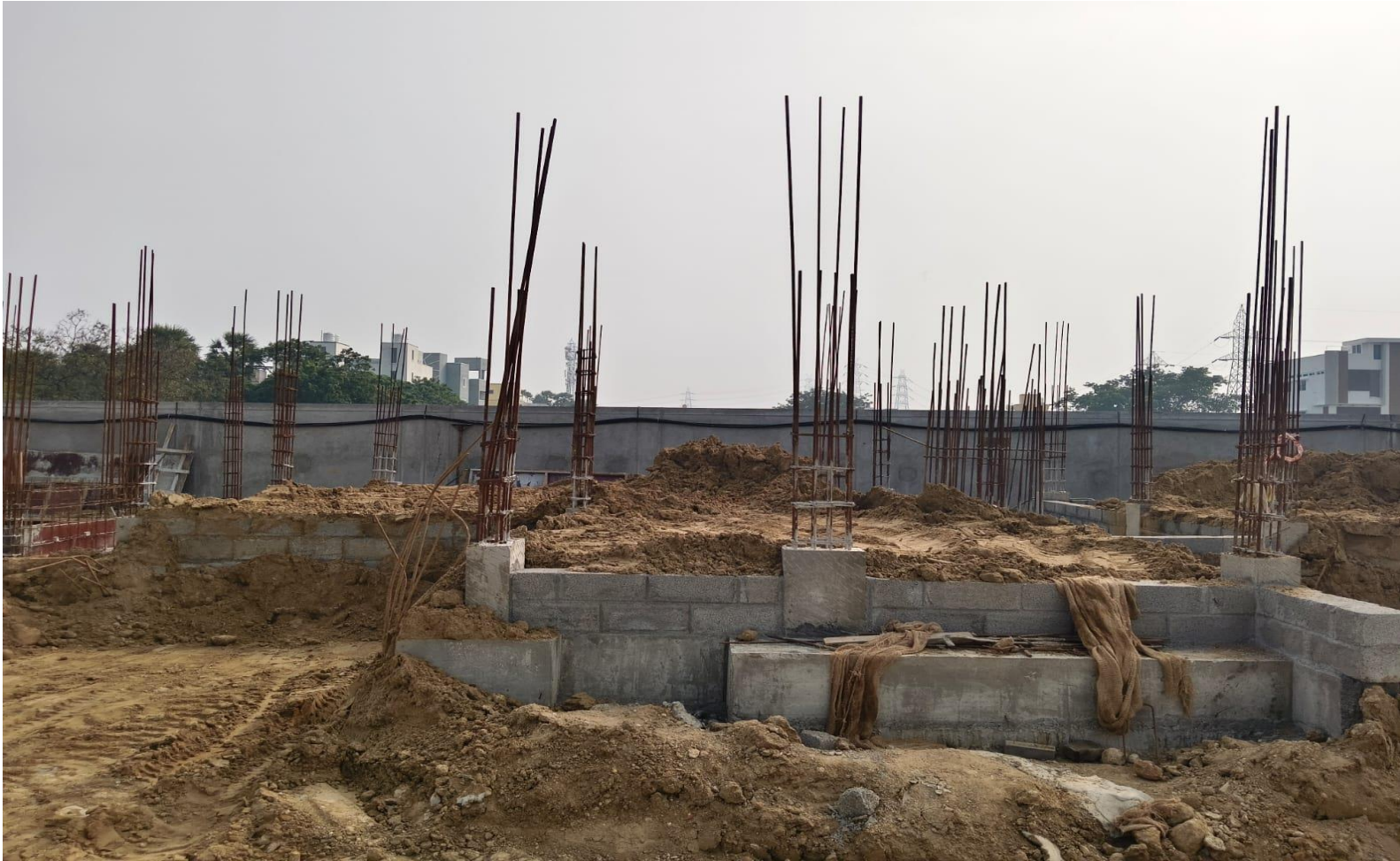
Villa No 25-Basement Back Filling Work In Progress
