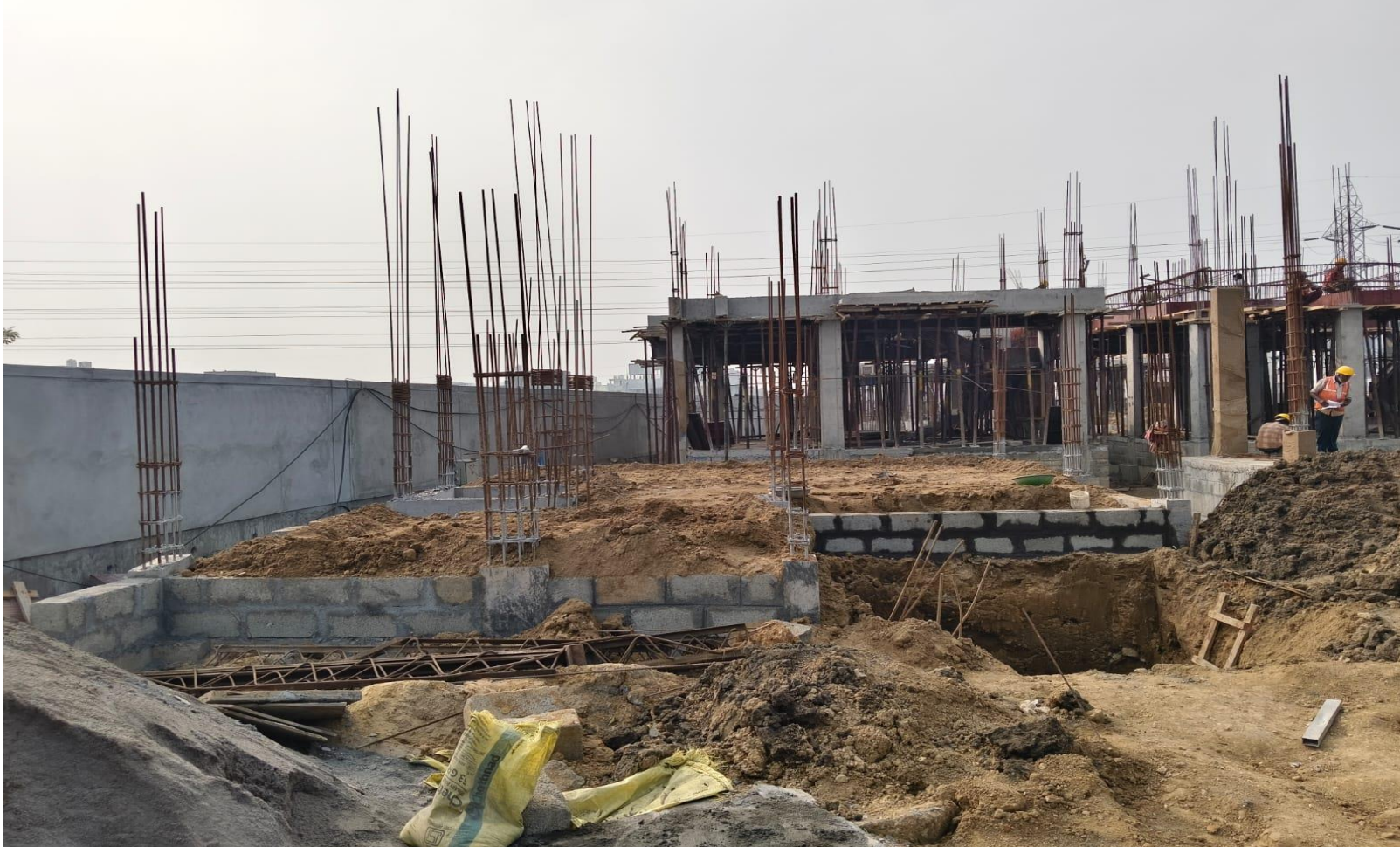
Villa No 30 - Basement Back Filling Work In Progress
