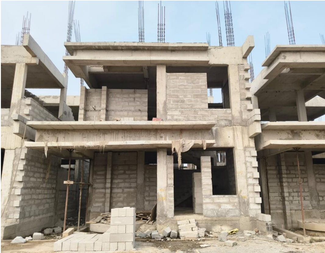
Villa - 49 -GF & FF Block Work In Progress
