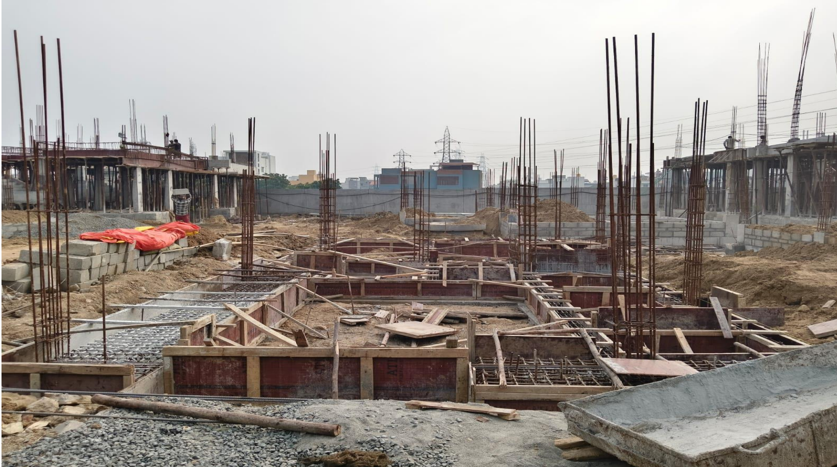
Villa No 41 –Plinth Beam Shuttering Work In Progress
