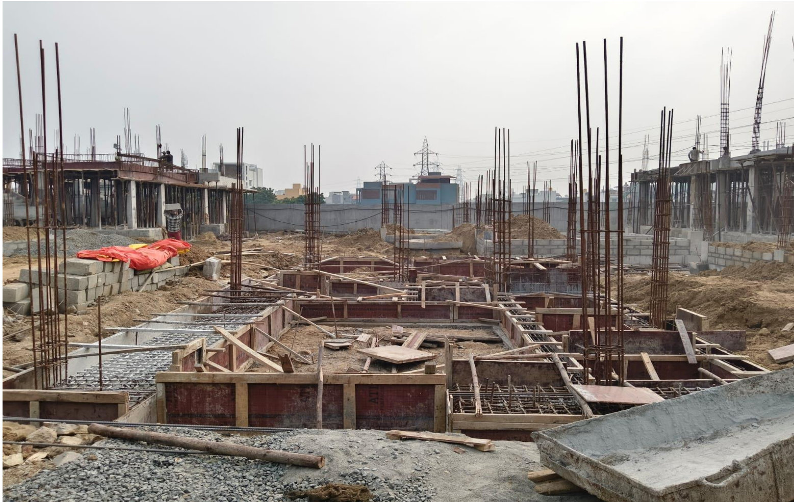
Villa No 41- Plinth Beam Shuttering work Completed
