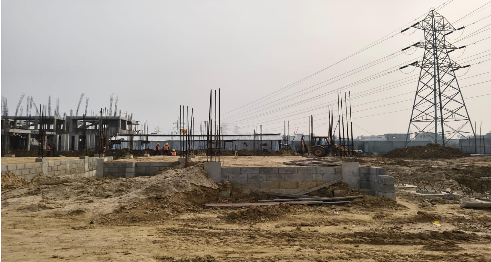
Villa No 81–Basement Back Filling Work Completed
