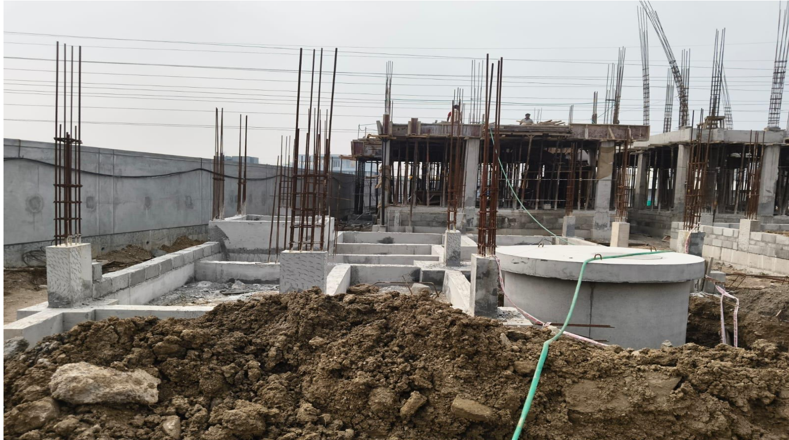
Villa No 39 –Plinth Beam Concrete Completed
