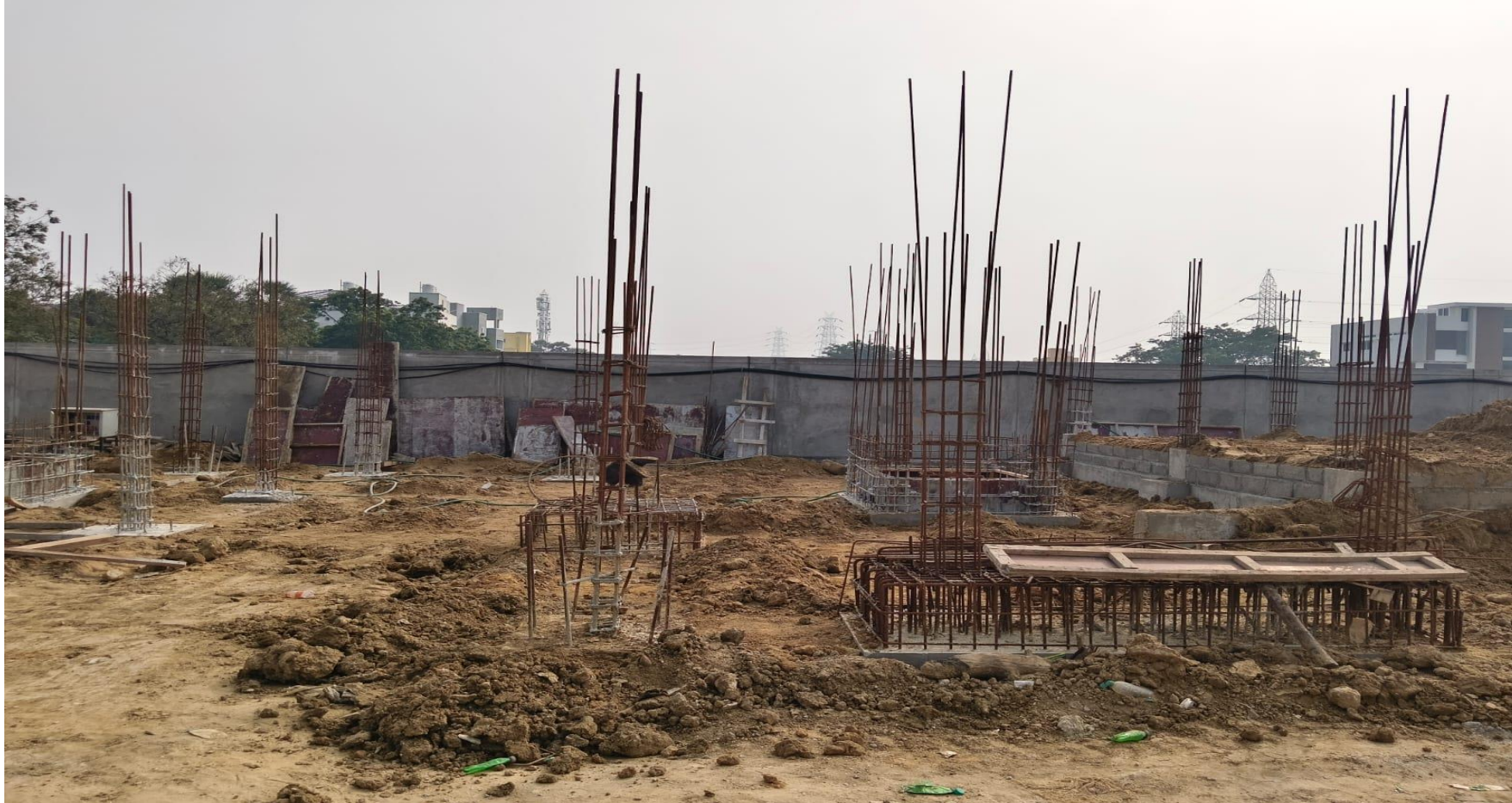
Villa No 24- Pile Cap Concrete work Completed
