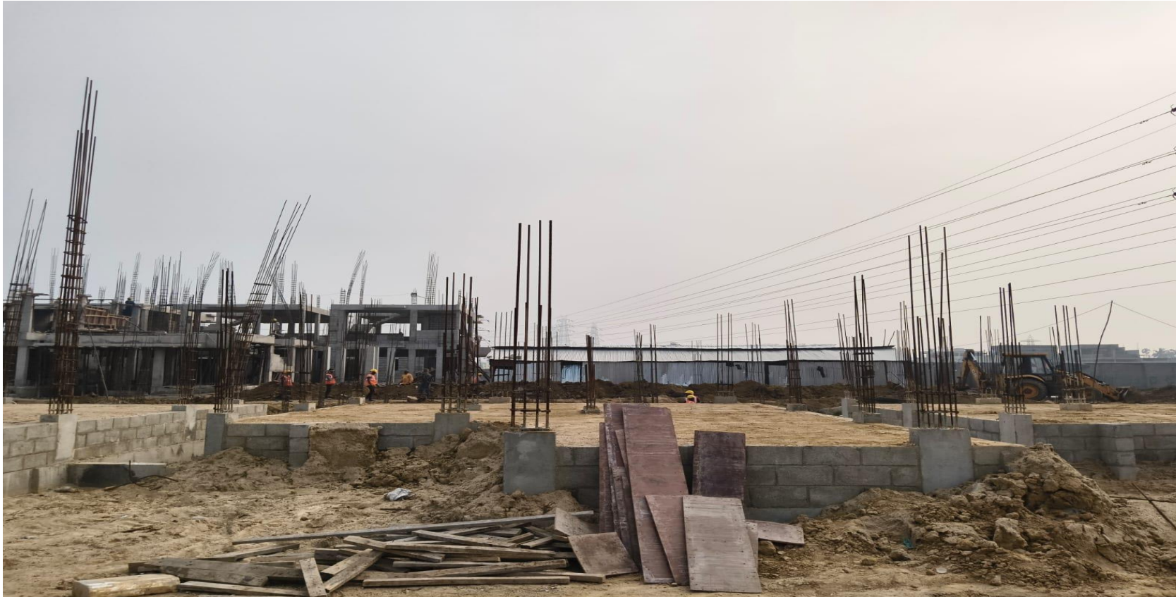
Villa No 80 –Basement Back Filling Work Completed
