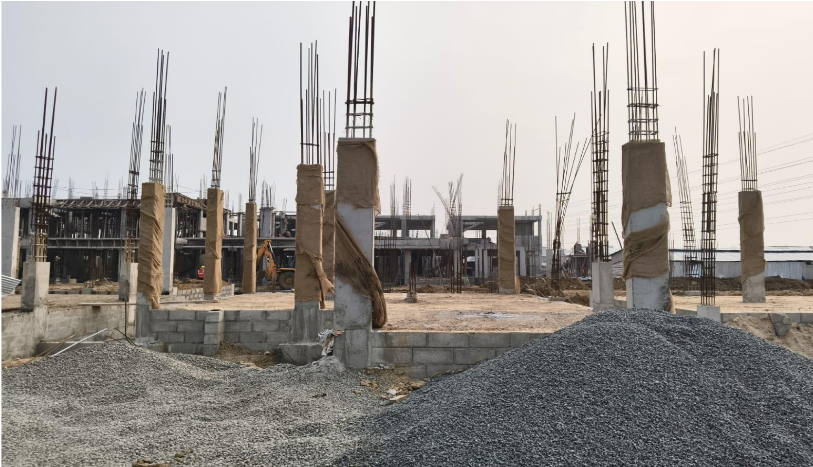
Villa No 78—GF column concrete completed
