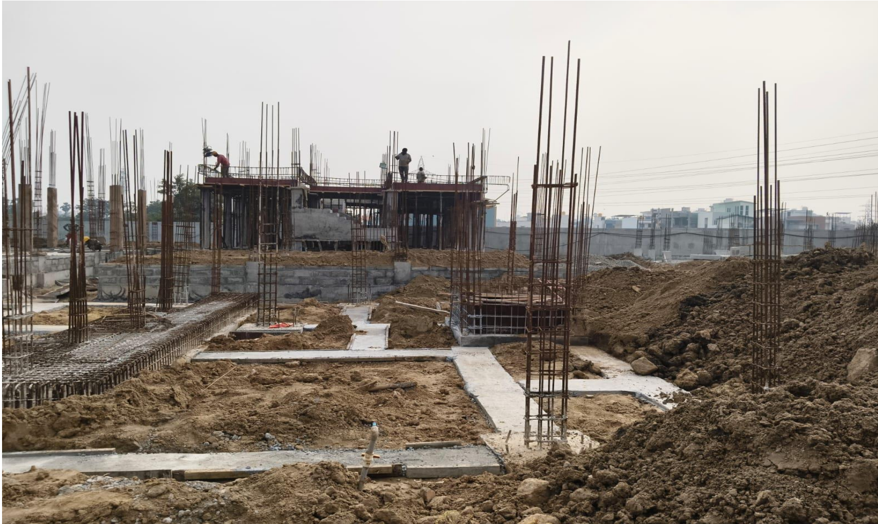
Villa No 35- Plinth Beam PCC work Completed
