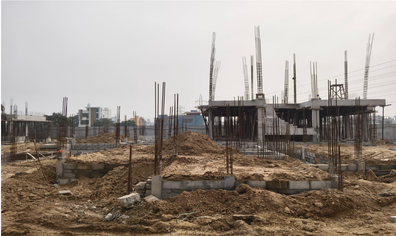
Villa No 42 –Basement Back Filling Work In Progress
