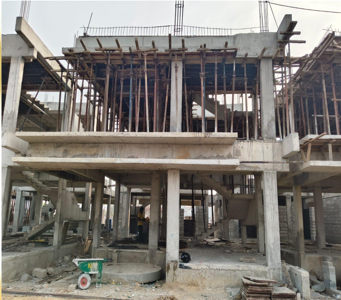
Villa - 57 - 1 st Floor Roof Slab Completed.
