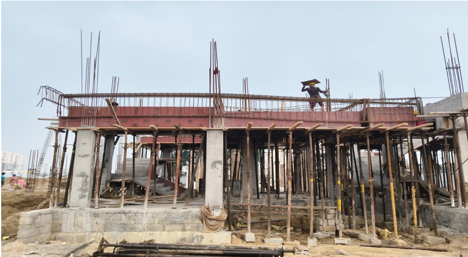
Villa No 37 –GF Roof Slab Reinforcement Work In Progress
