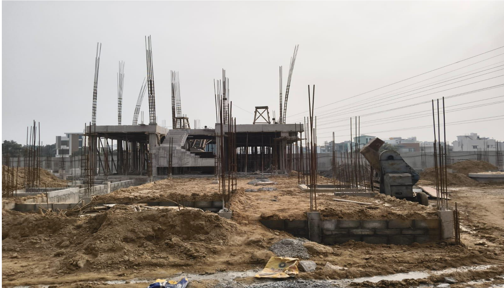
Villa No 43- Basement Back Filling work Completed
