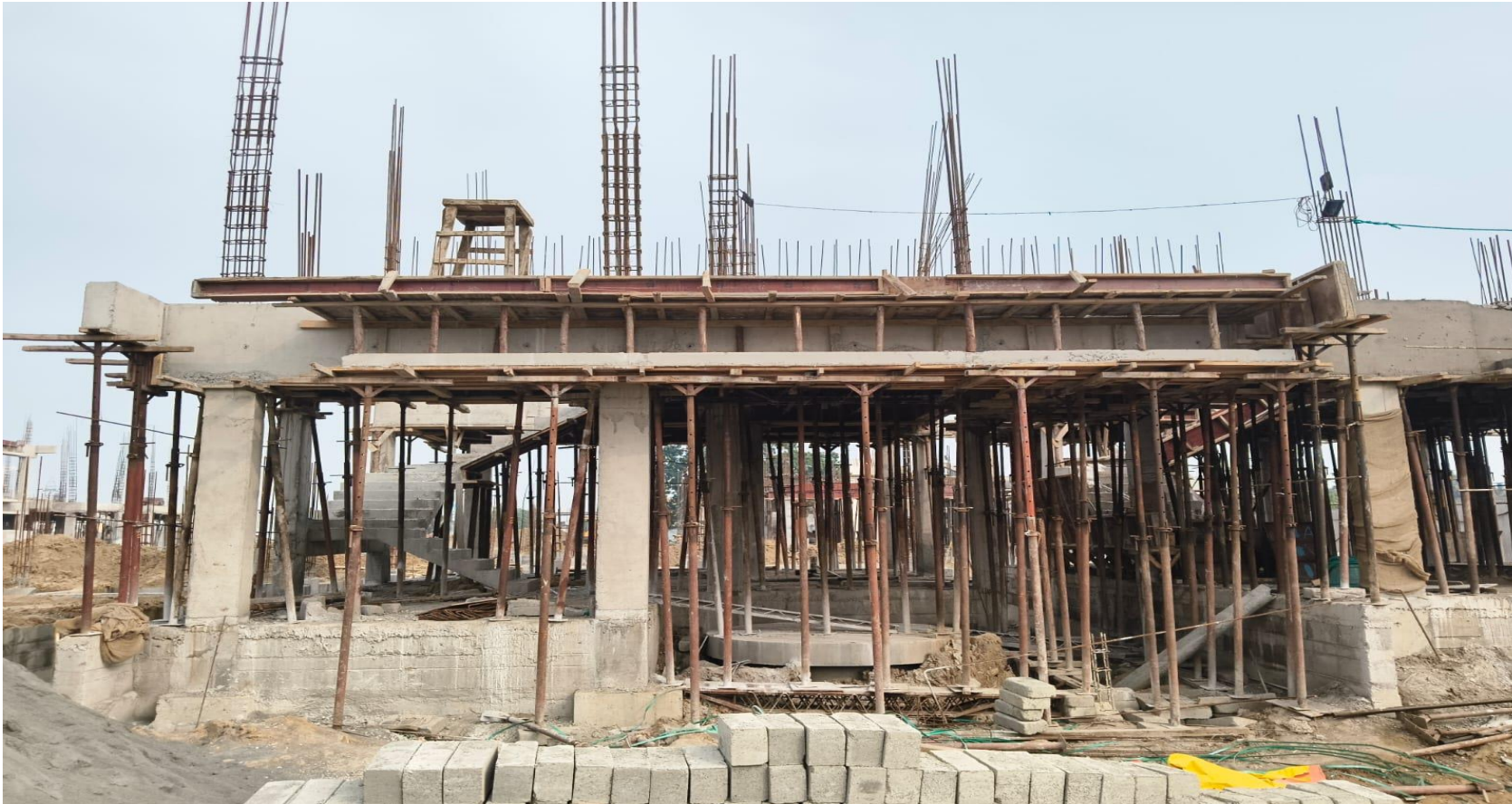
Villa No 44–FF Column Reinforcement Work Completed
