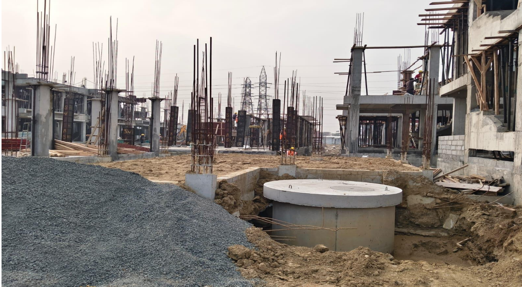
Villa No 72 –Basement Back Filling Work In Progress
