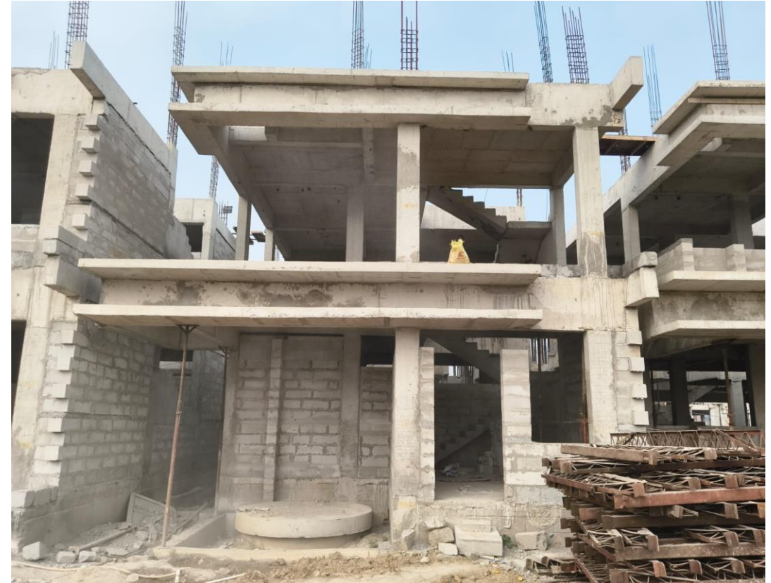
Villa - 50 -GF Block Work In Progress
