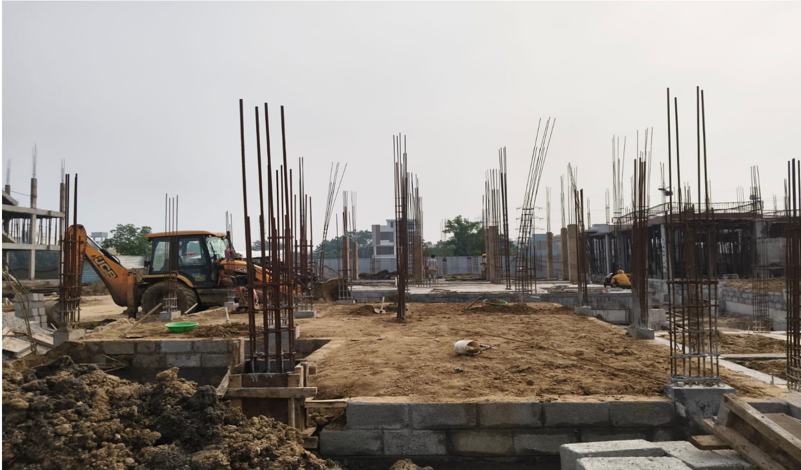
Villa No 33- Basement Back Filling Work In Progress
