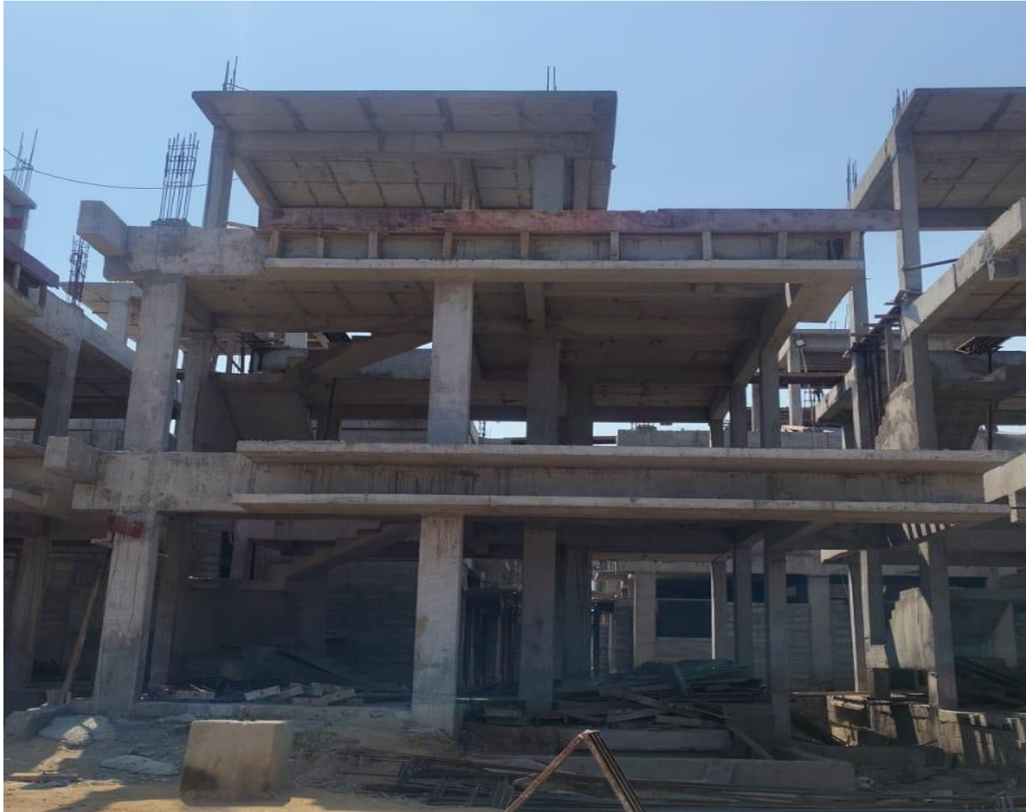
Villa No 54 – Head Room Roof Salb Concrete Pouring Completed
