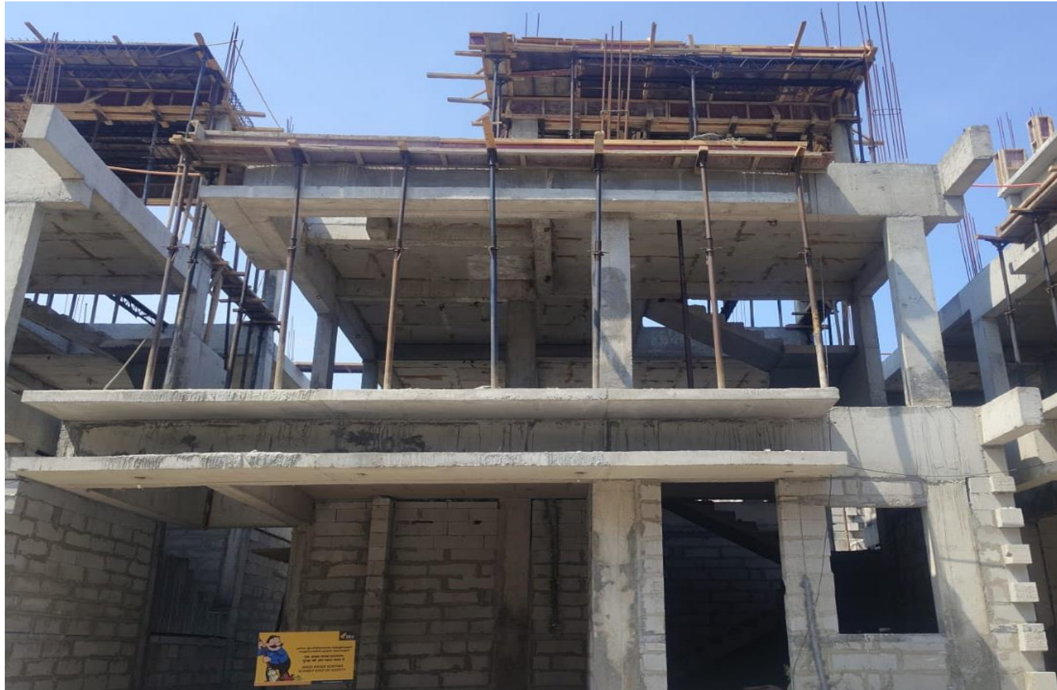
Villa No 68–Head Room Roof Slab Concrete Pouring Completed
