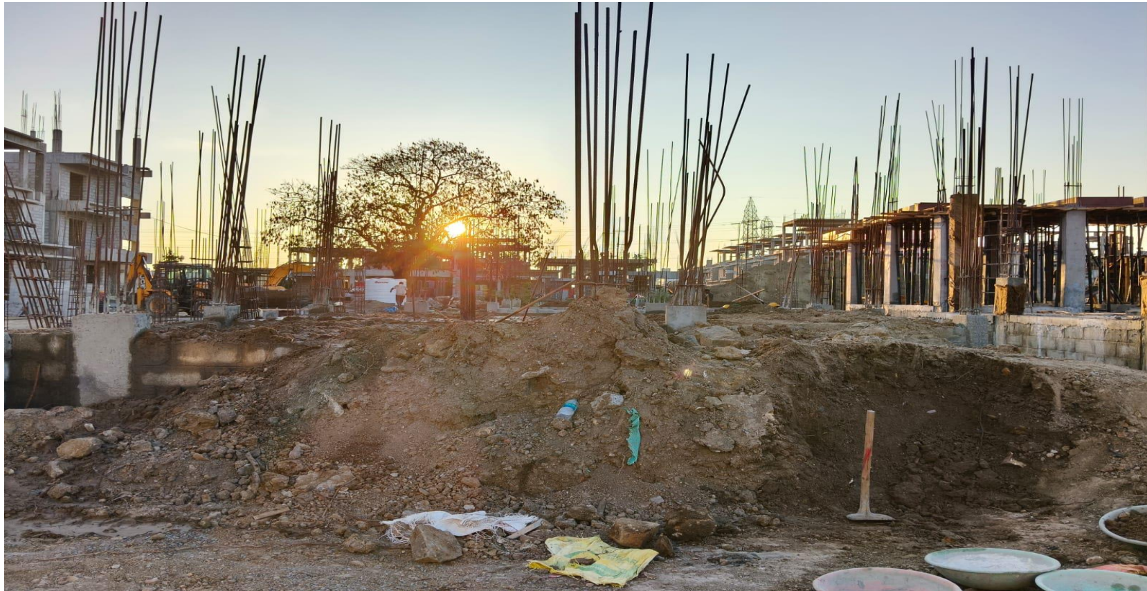
Villa No 118–Basement Back Filling Work Completed
