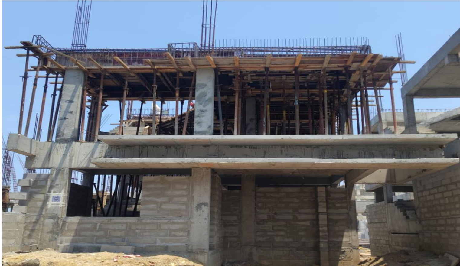
Villa No 37 –FF Roof Slab Reinforcement Work In Progress
