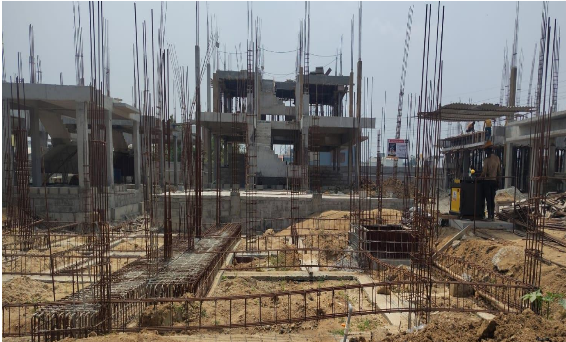
Villa No 35- Plinth Beam Reinforcement work Completed
