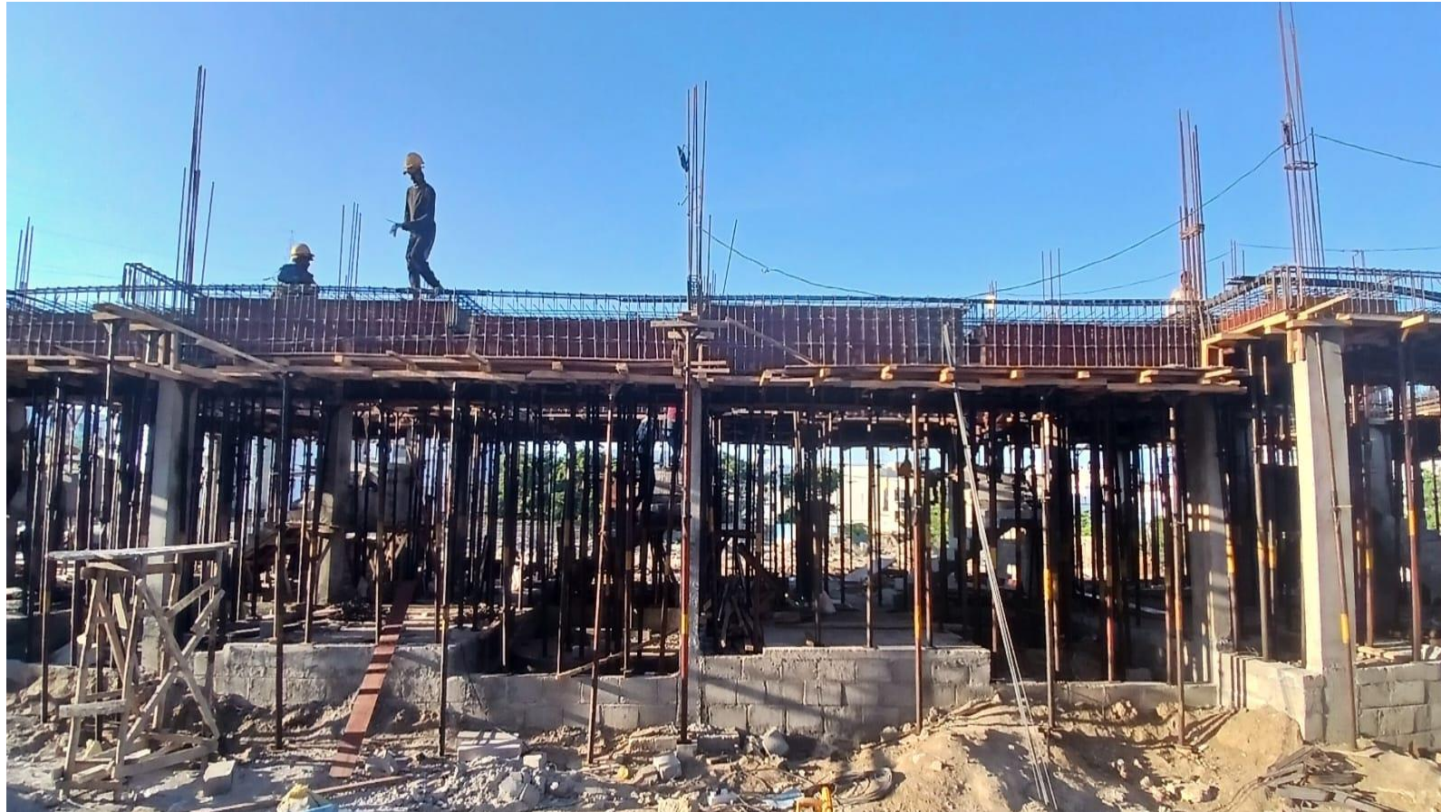
Villa No 94 to 98–GF Roof Slab Shuttering Work In Progress
