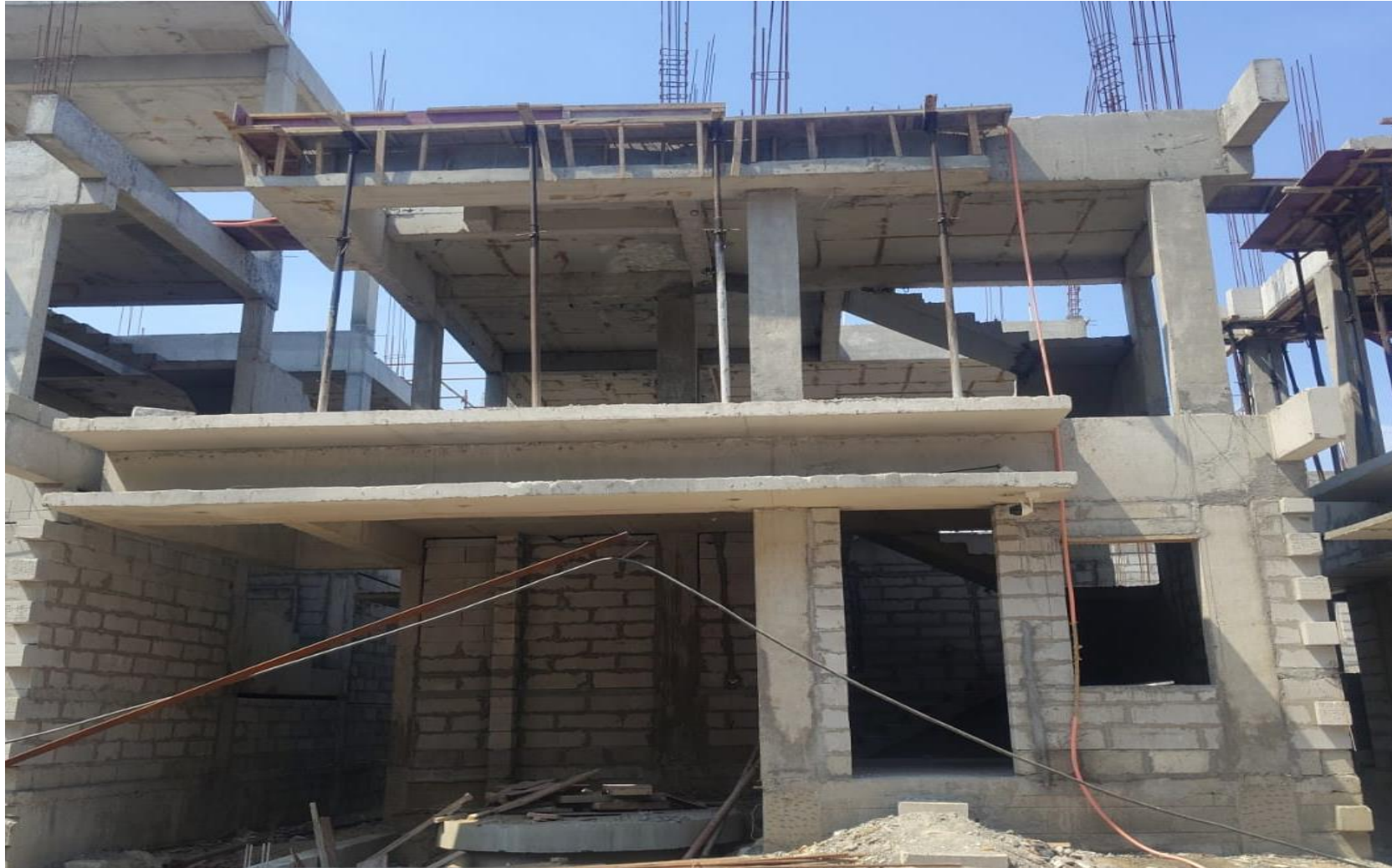
Villa No 70–SF Column Reinforcement Work In Progress
