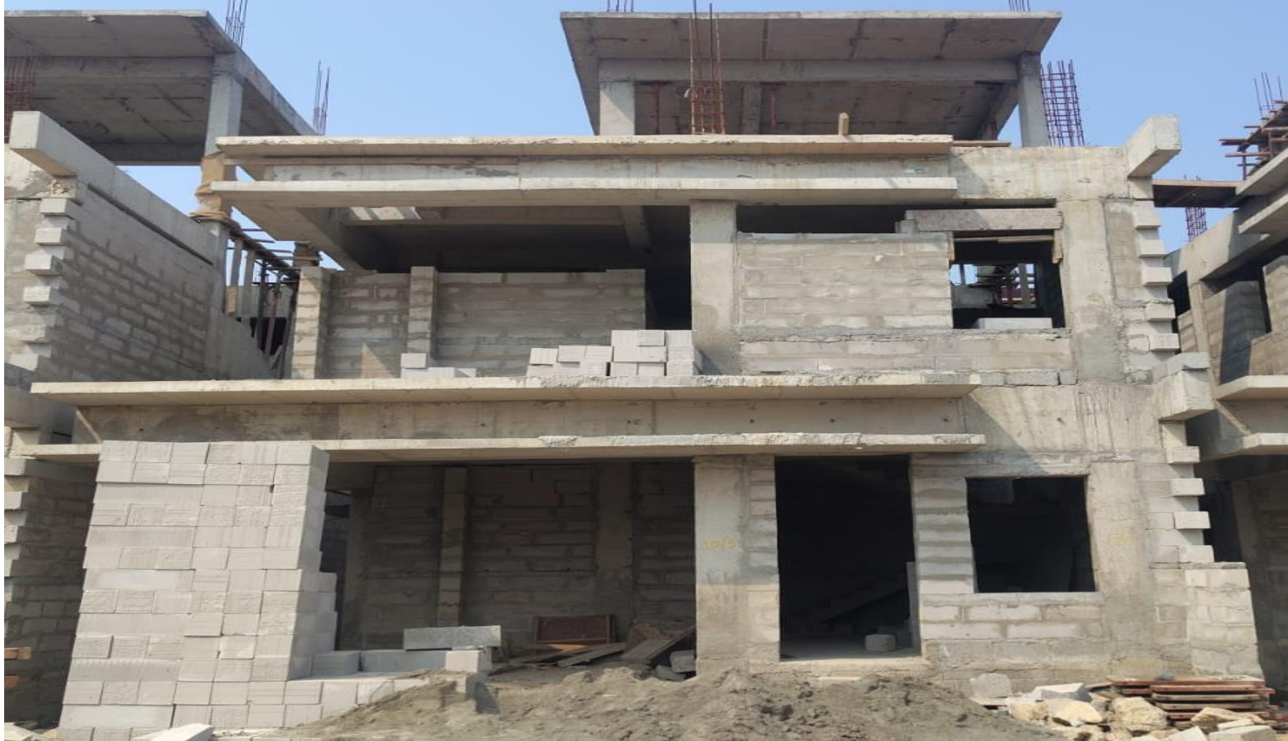
Villa No -51 GF&FF Block Work In Progress
