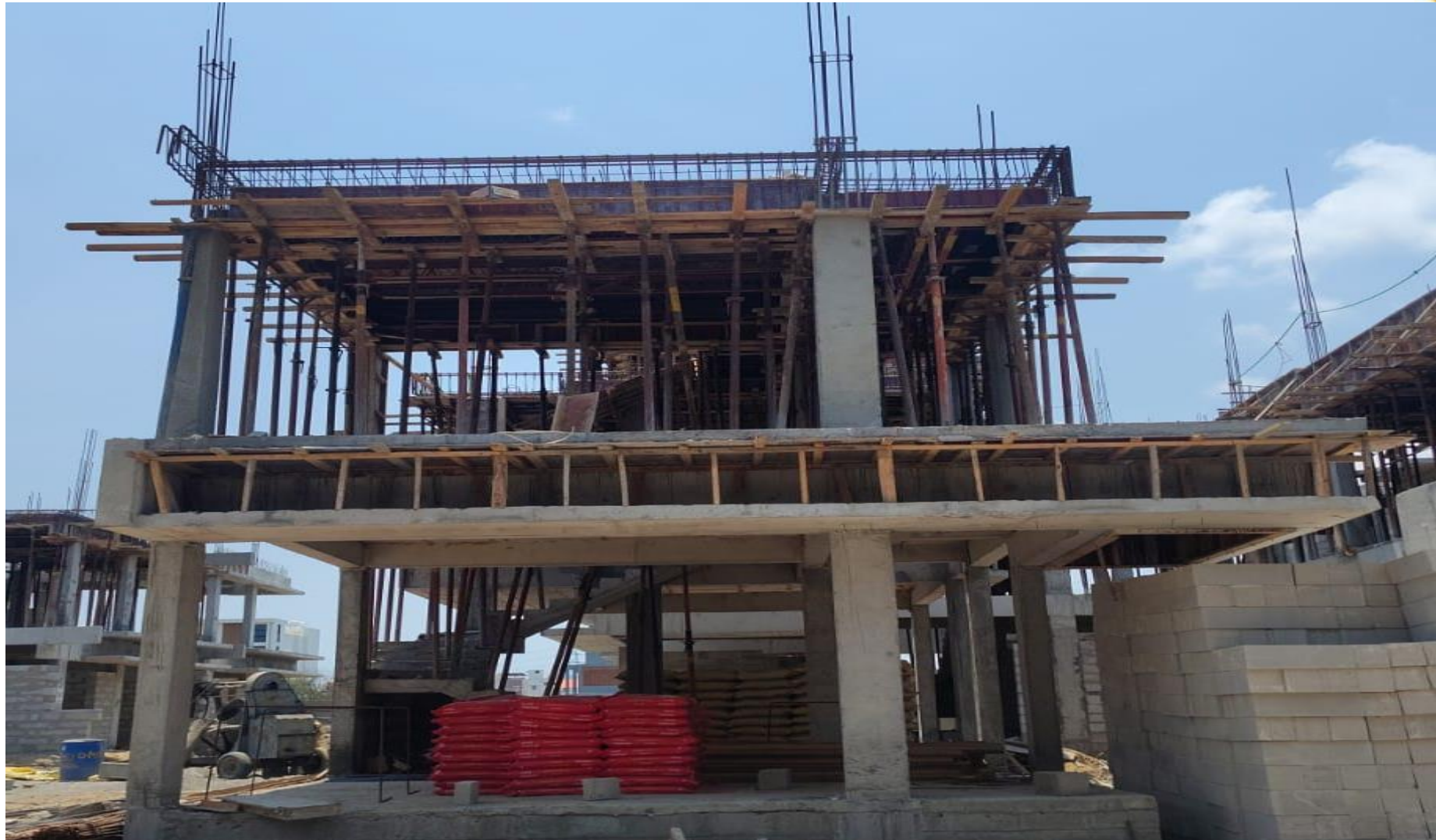
Villa No 41- FF Roof Slab Reinforcement work Progress
