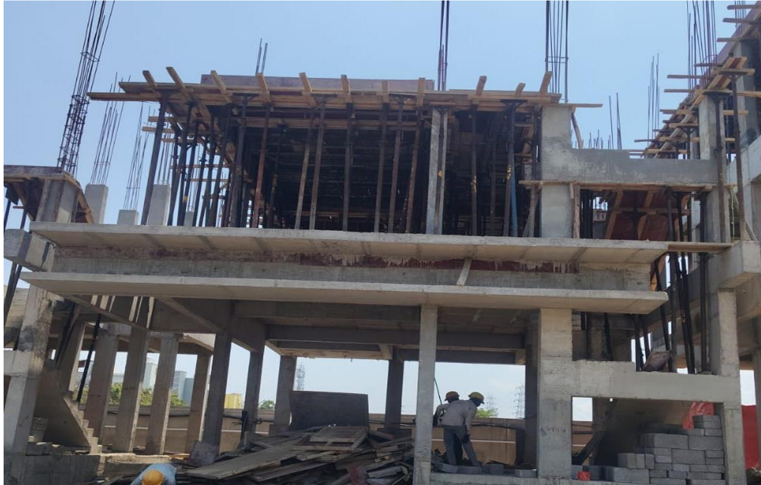
Villa No 26- FF Roof Slab Shuttering Work In Progress
