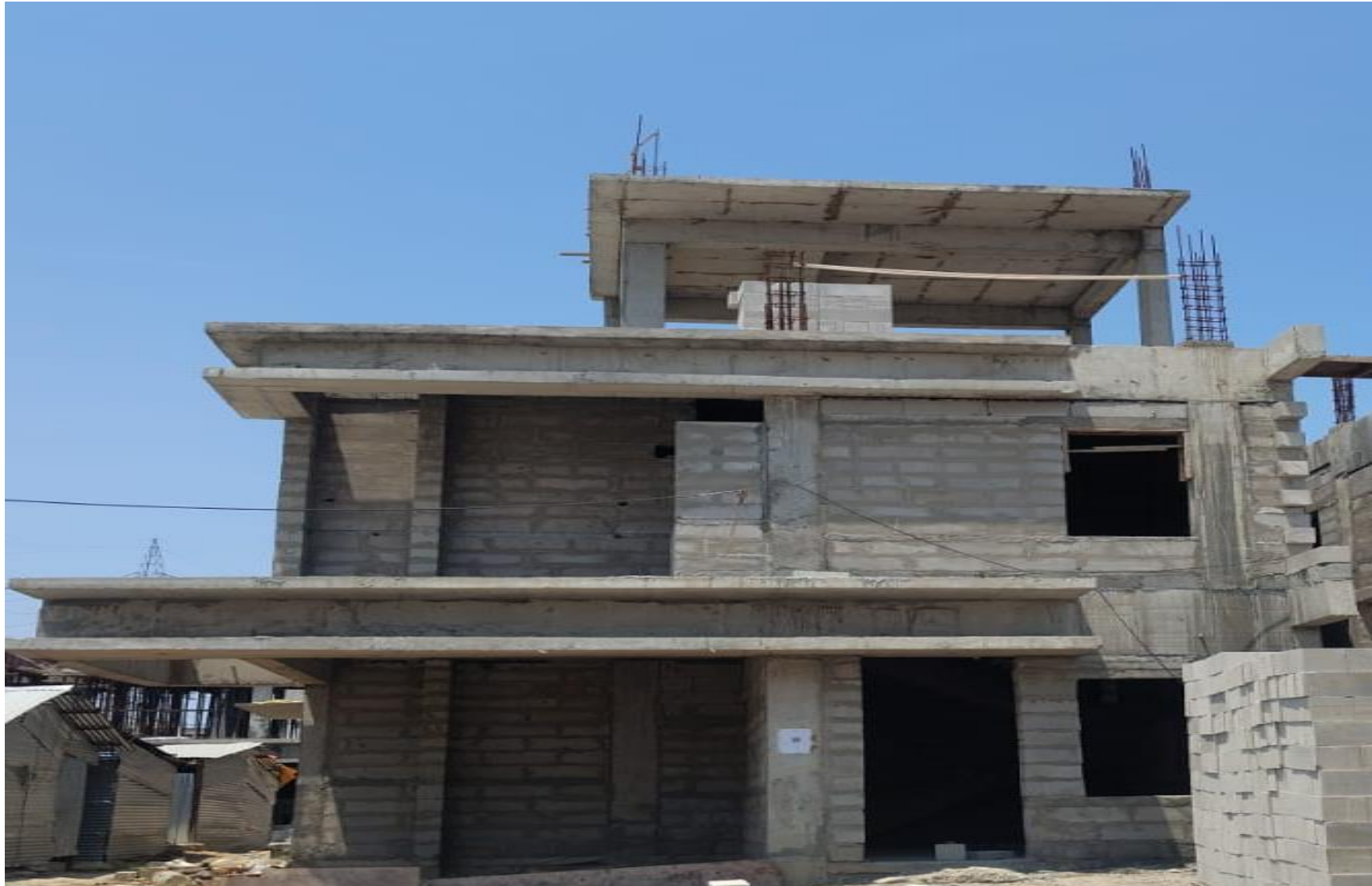
Villa No 47 –Head Room Slab Concrete Pouring Completed
