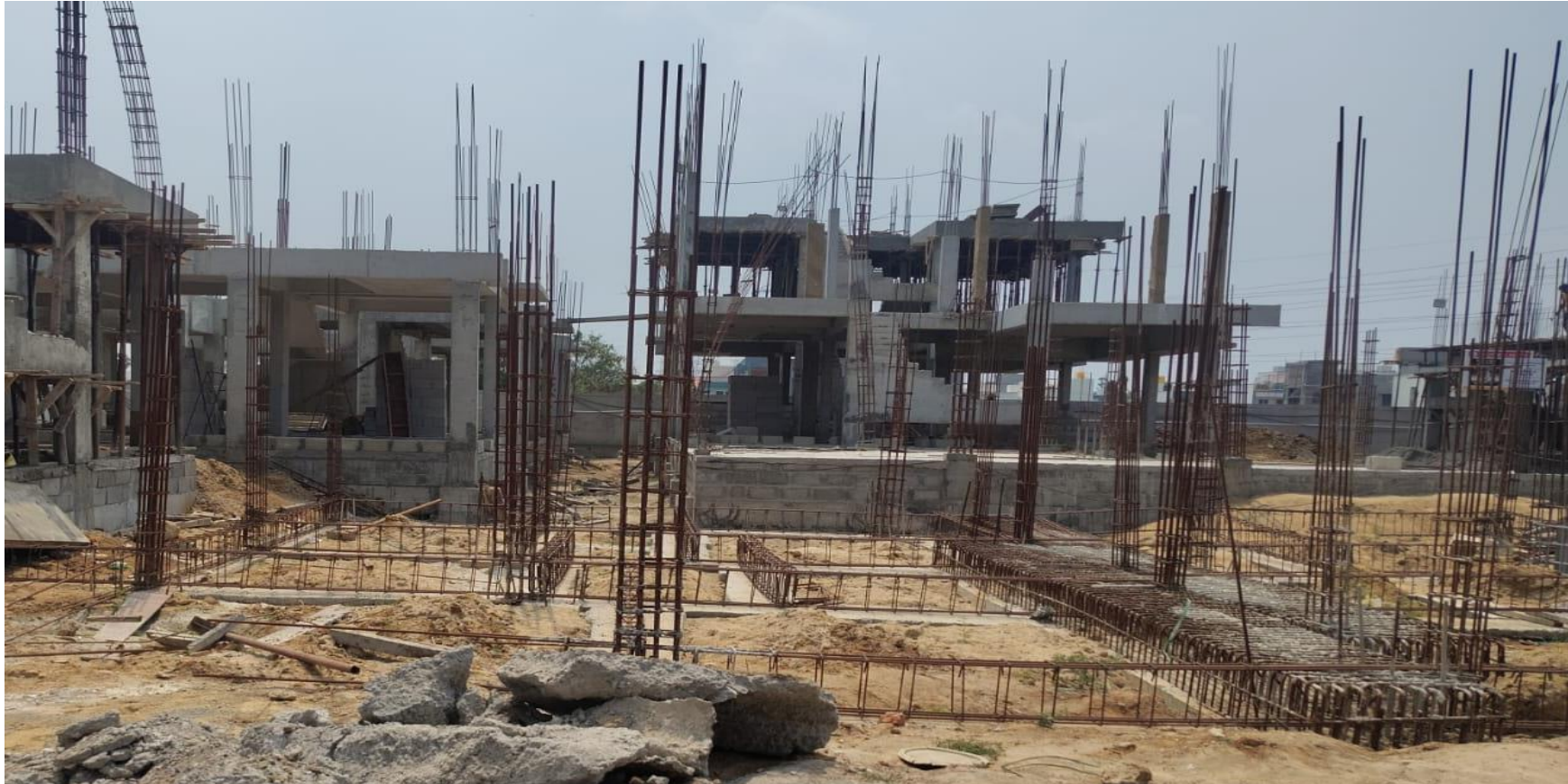
Villa No 34 – Plinth Beam Reinforcement Work In Progress
