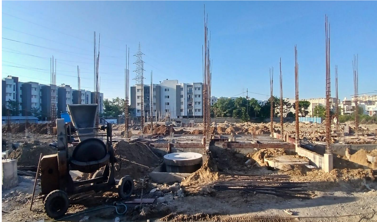
Villa No 90 & 91–GF Column Reinforcement Work In Progress
