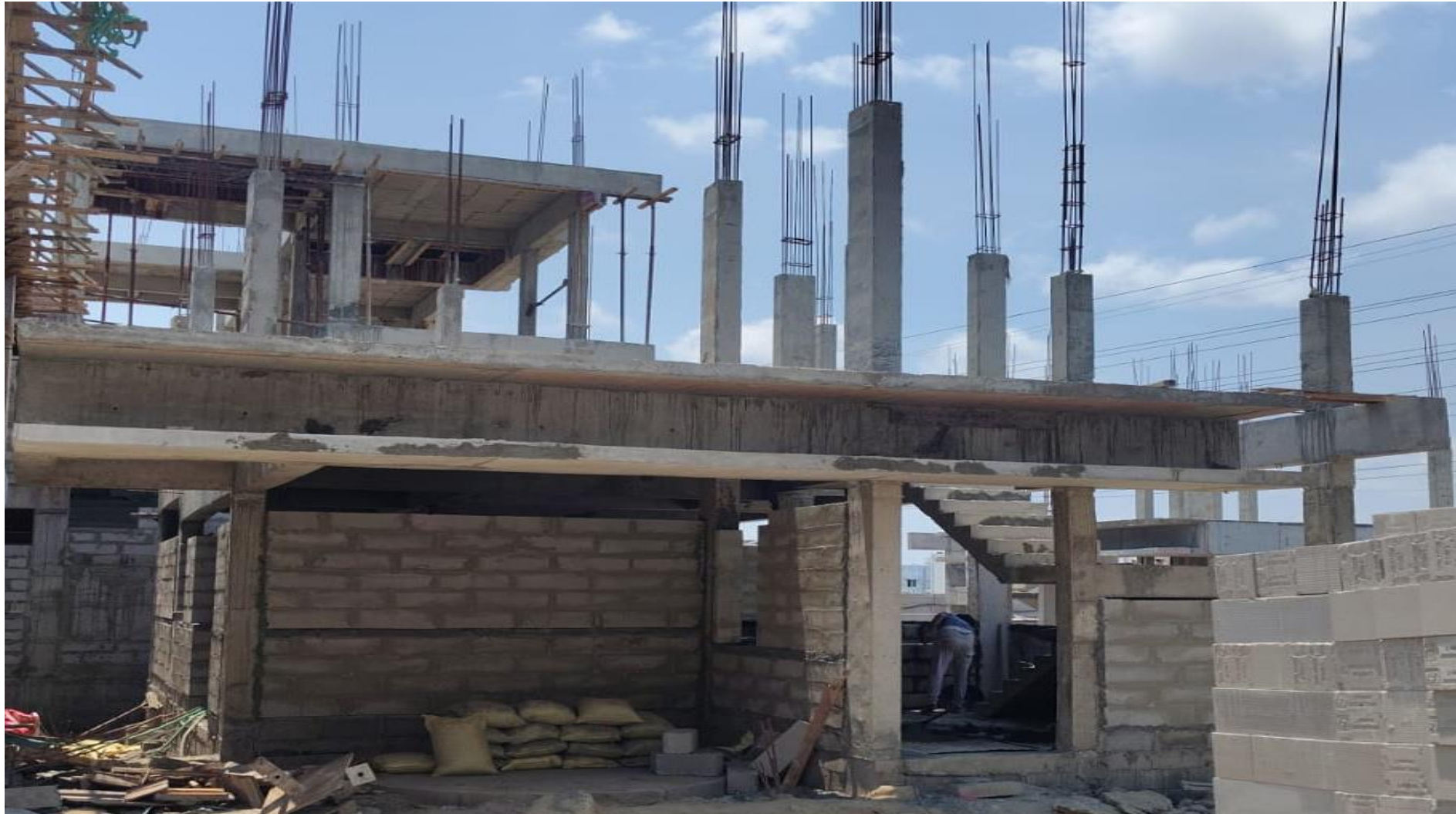
Villa No 43- FF Column Concrete Work Completed
