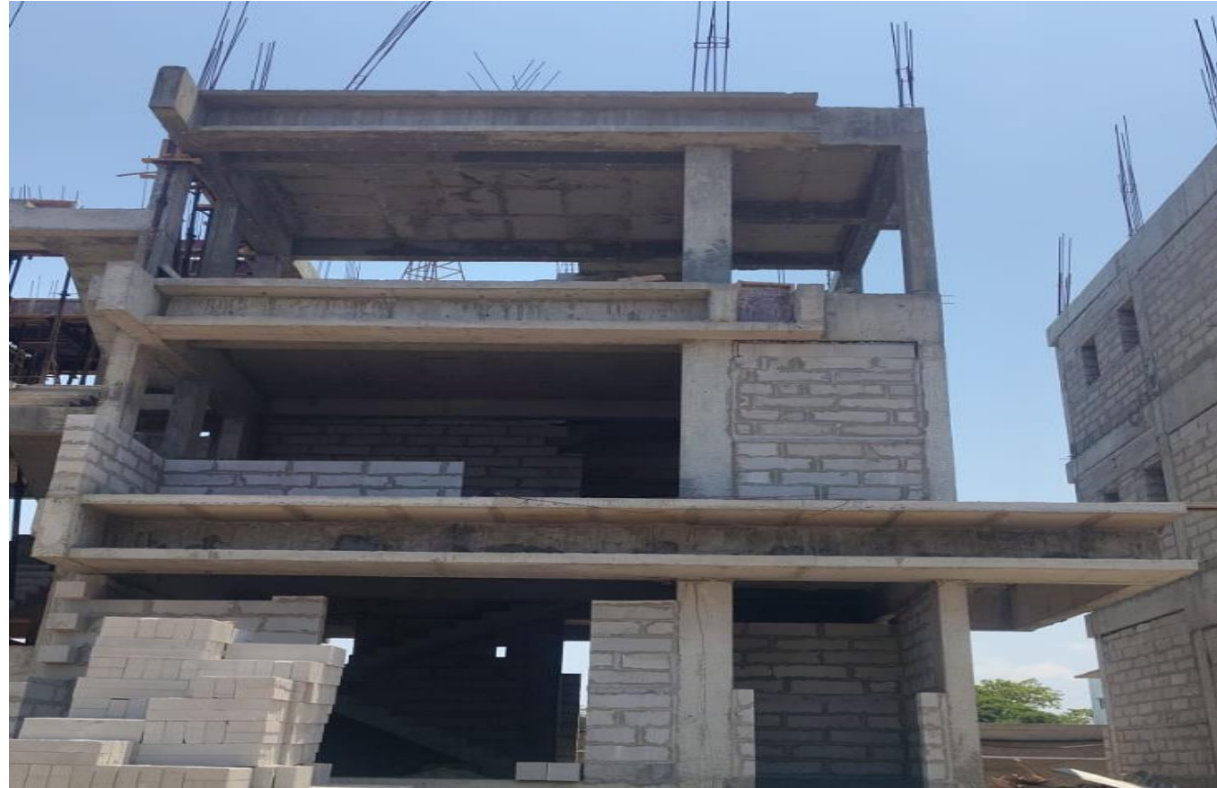
Villa No 28 –FF Block Work In Progress
