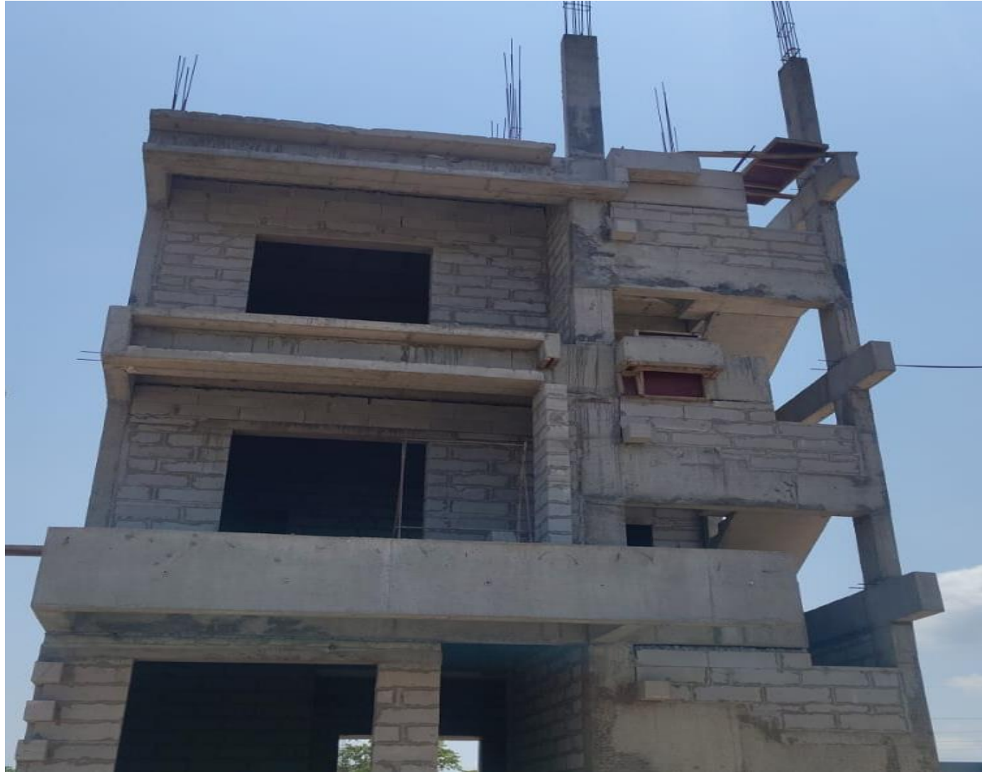
Villa No-29 Head Room Column Concrete work Completed
