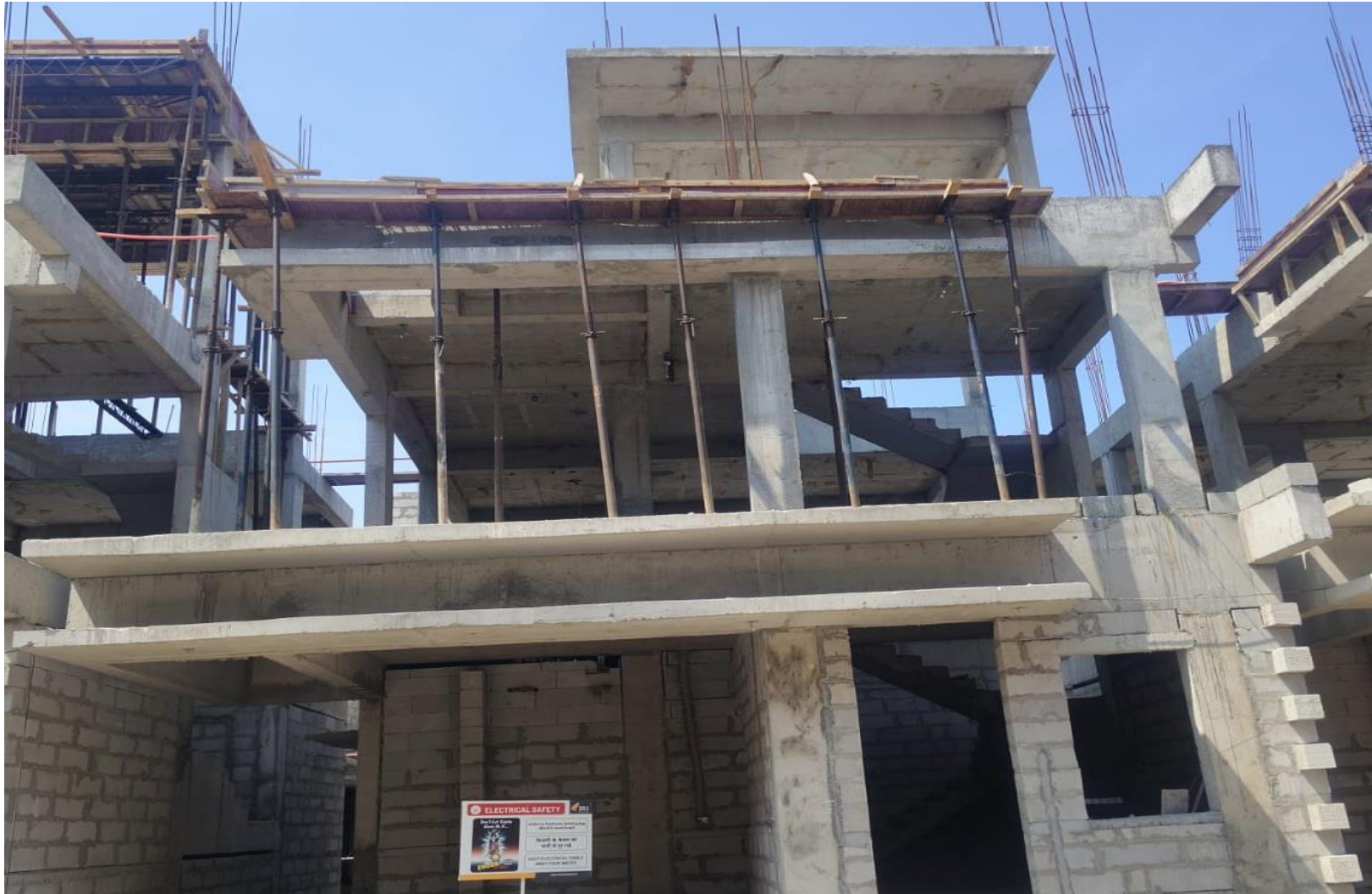
Villa No 69 –Head Room Roof Slab Concrete Pouring Work Completed
