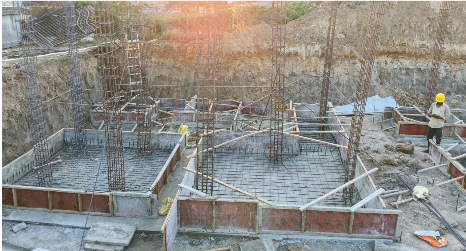
Villa No 110–Footing Shuttering Work In Progress
