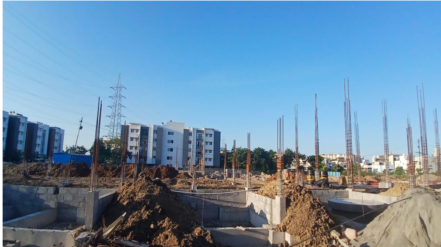
Villa No 87–Basement Backfilling Work In Progress
