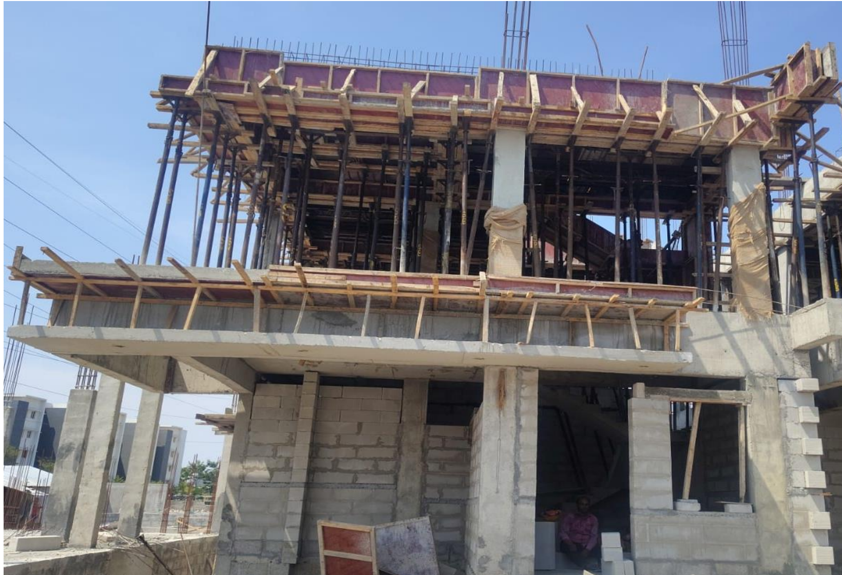
Villa No –63 FF Roof Slab Concrete Pouring Completed
