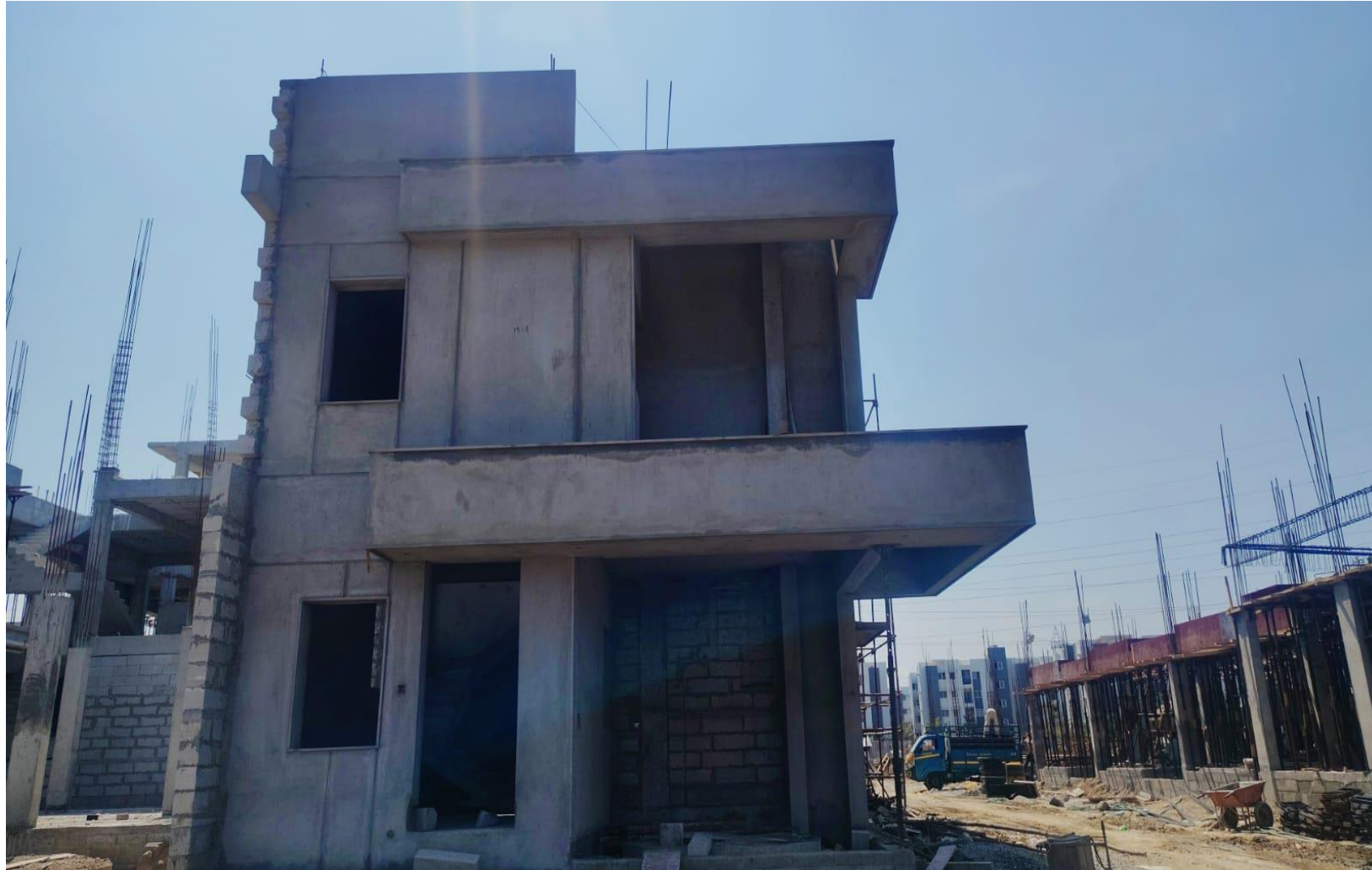
Villa No 73 – External Plastering Work In Progress
