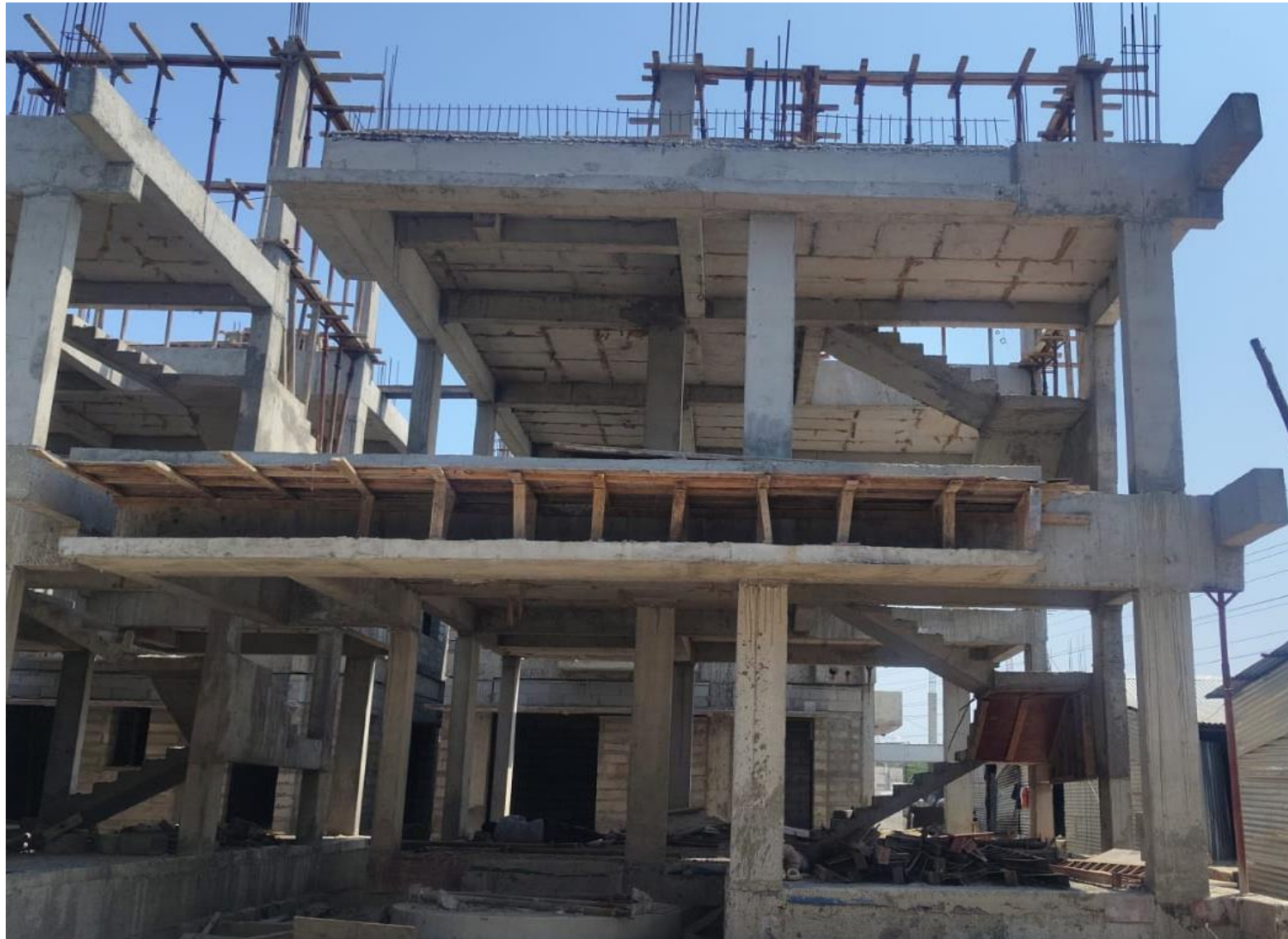
Villa No 61 –Head Room Roof Slab Shuttering Work In Progress
