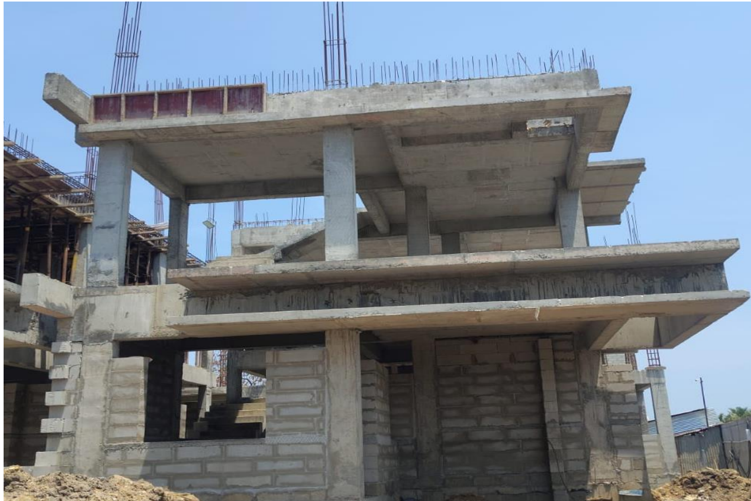
Villa No 38–GF Block Work In Progress
