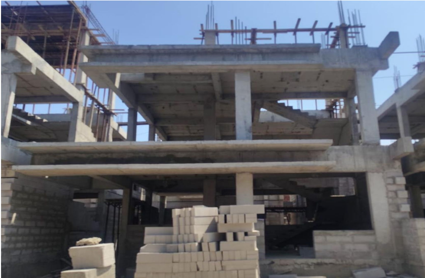
Villa No 59 –Head Room Roof Slab Shuttering Work In Progress
