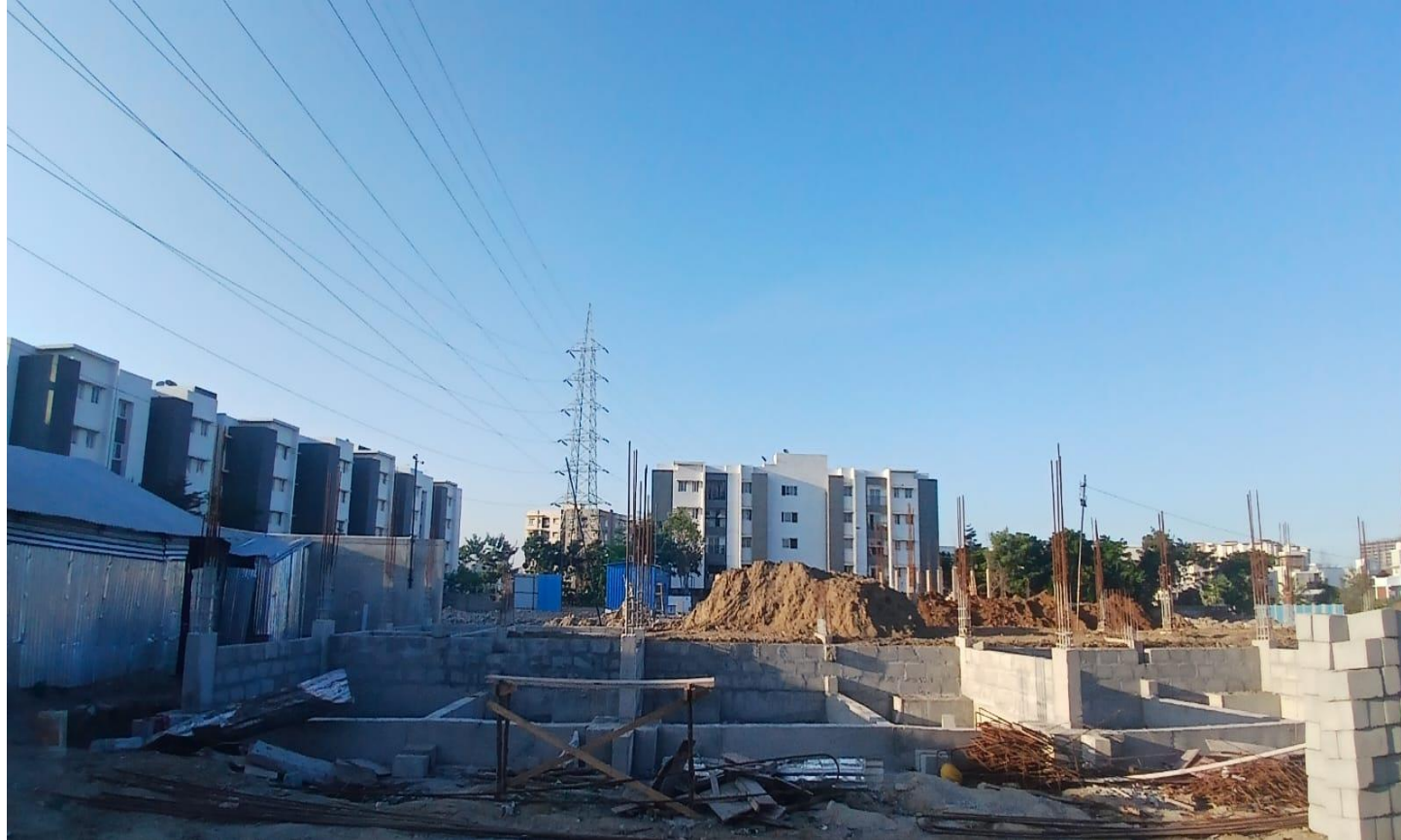
Villa No 83 & 84–Basement Block Work In Progress
