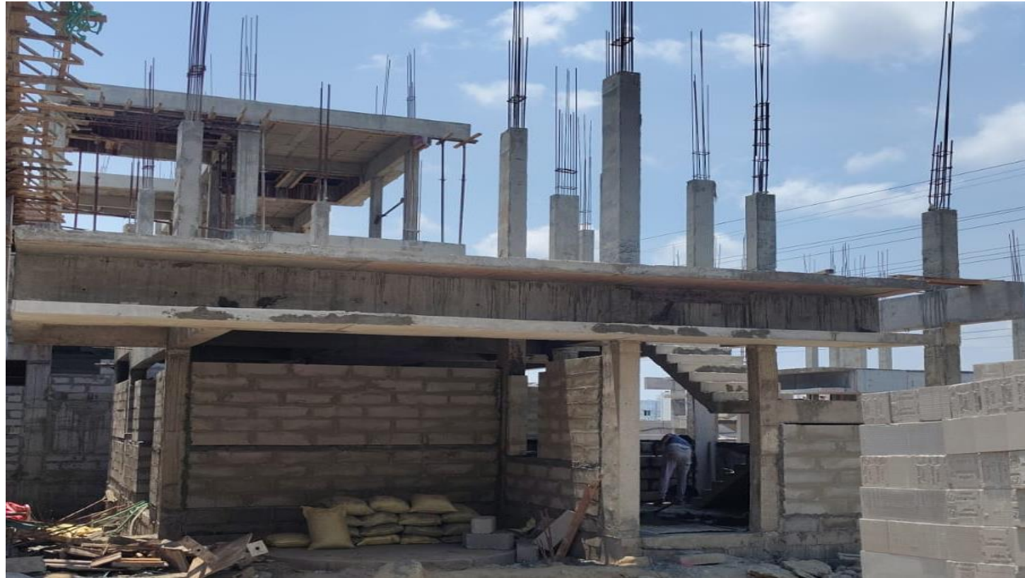
Villa No 43- FF Column Concrete Work Completed
