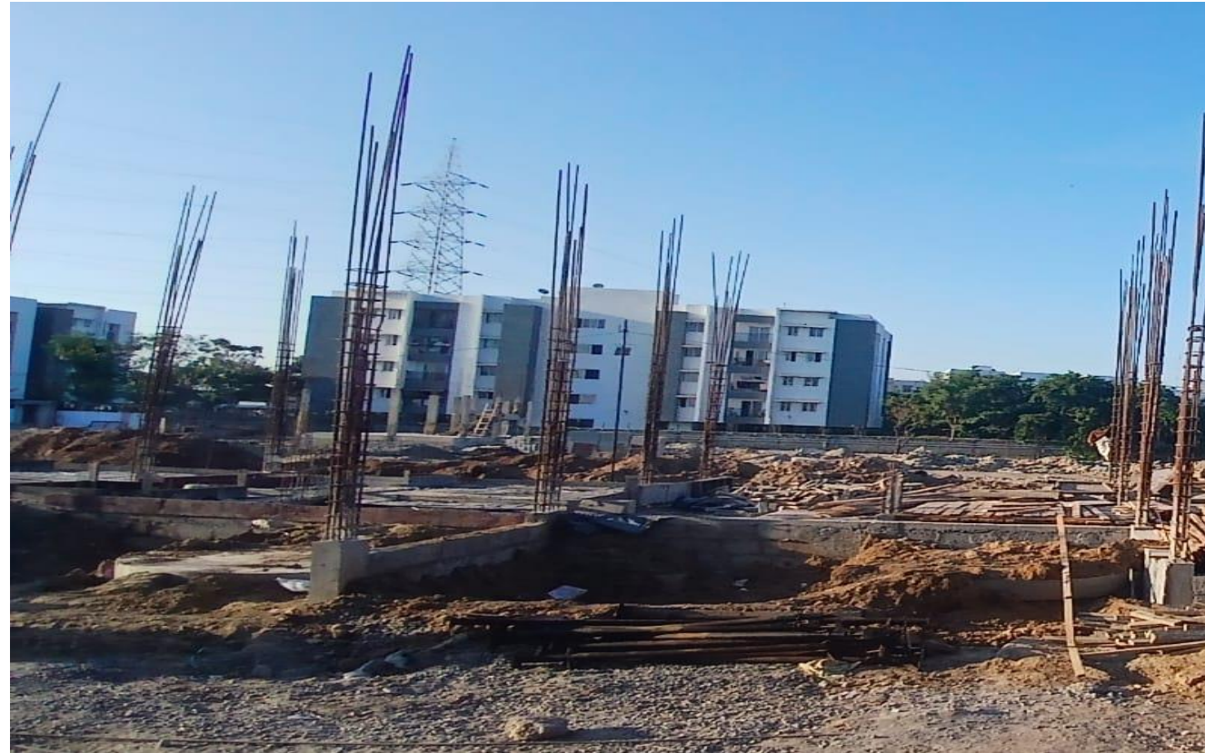
Villa No 92&93–GF Column Reinforcement Work In Progress
