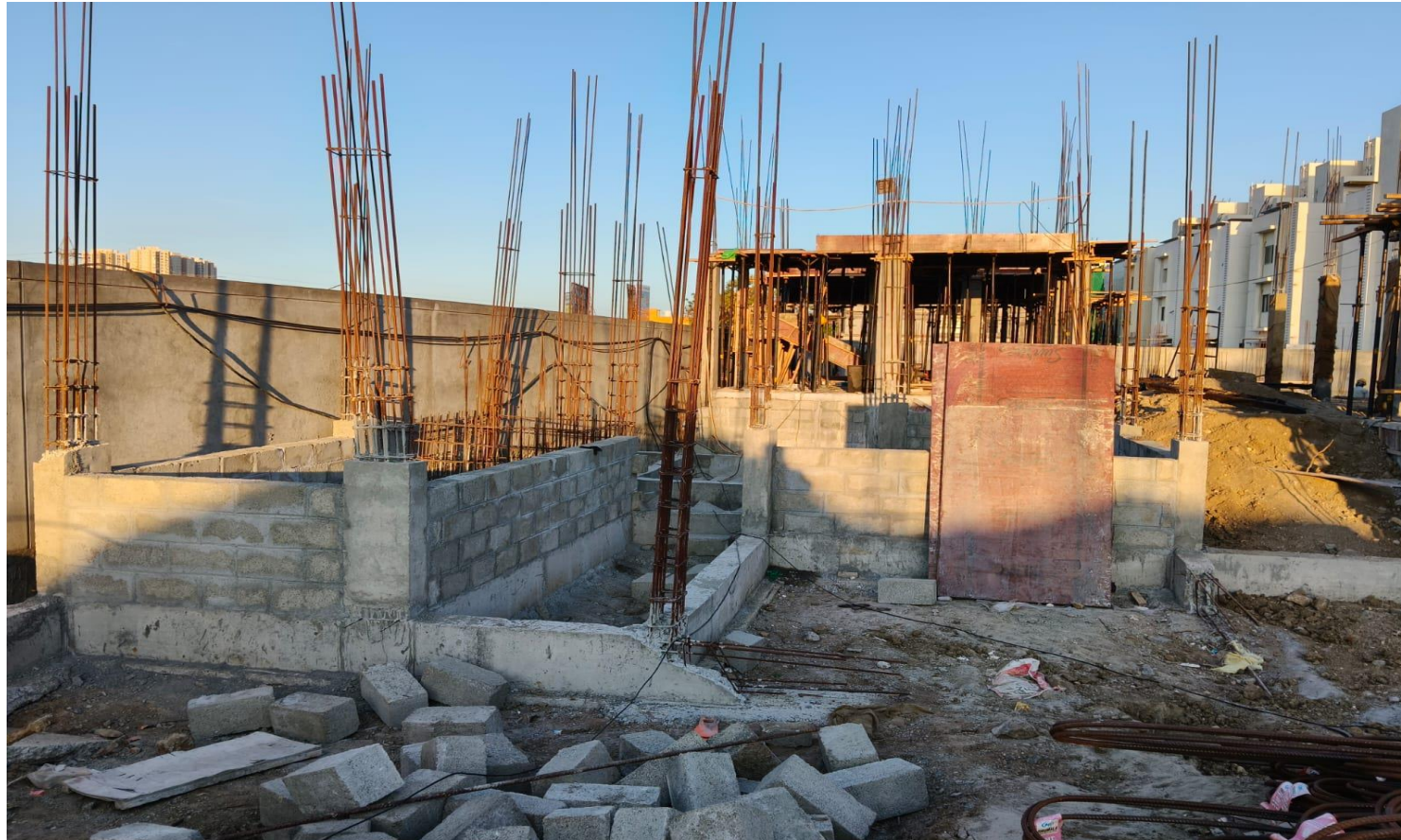
Villa No 113–Basement Block Work Completed
