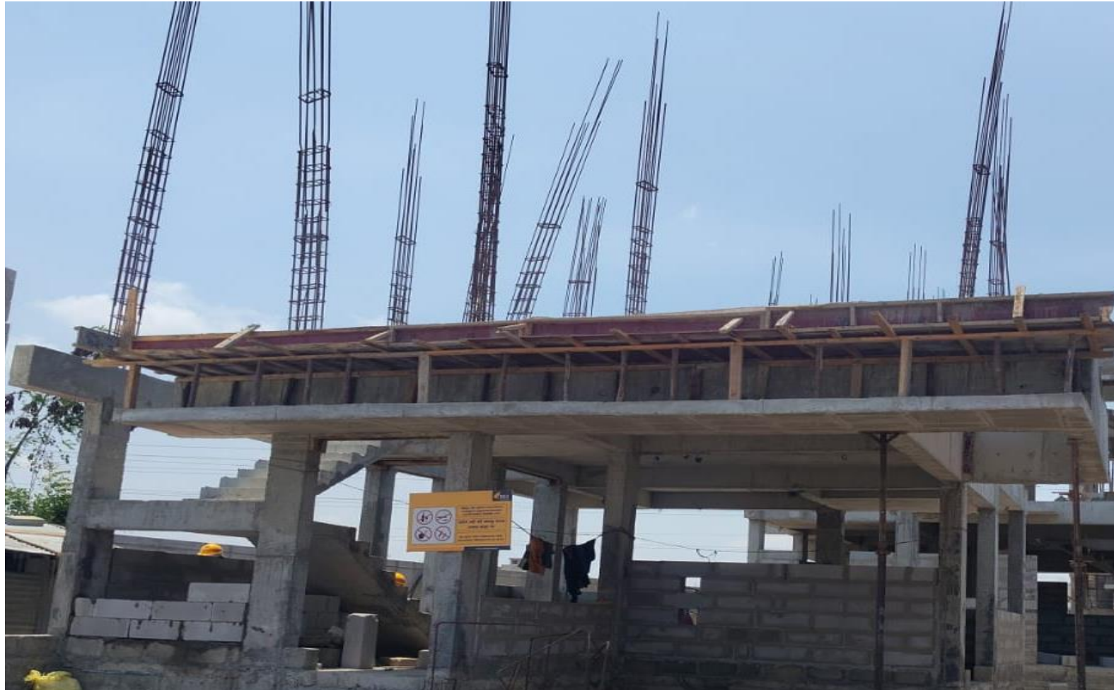
Villa No 30 – GF Block Work In Progress
