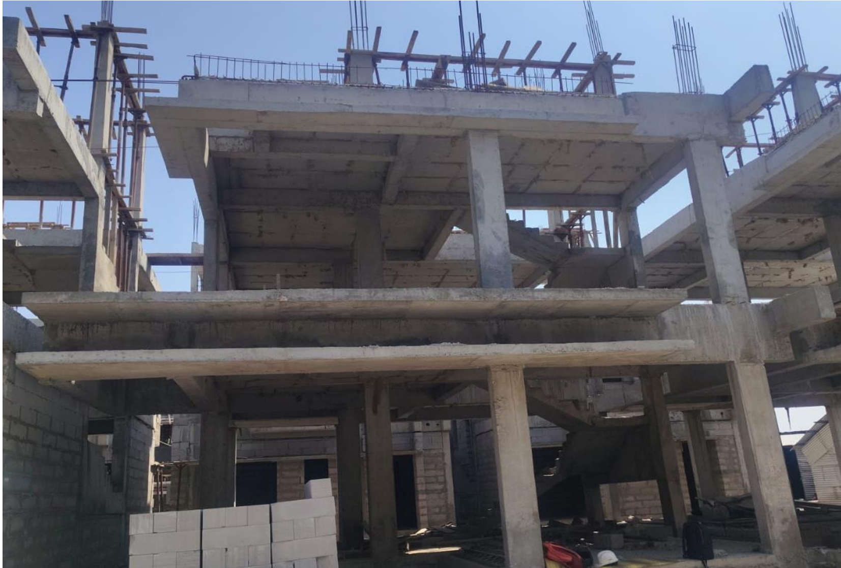
Villa No 60 – Head Room Roof Slab Shuttering Work In Progress
