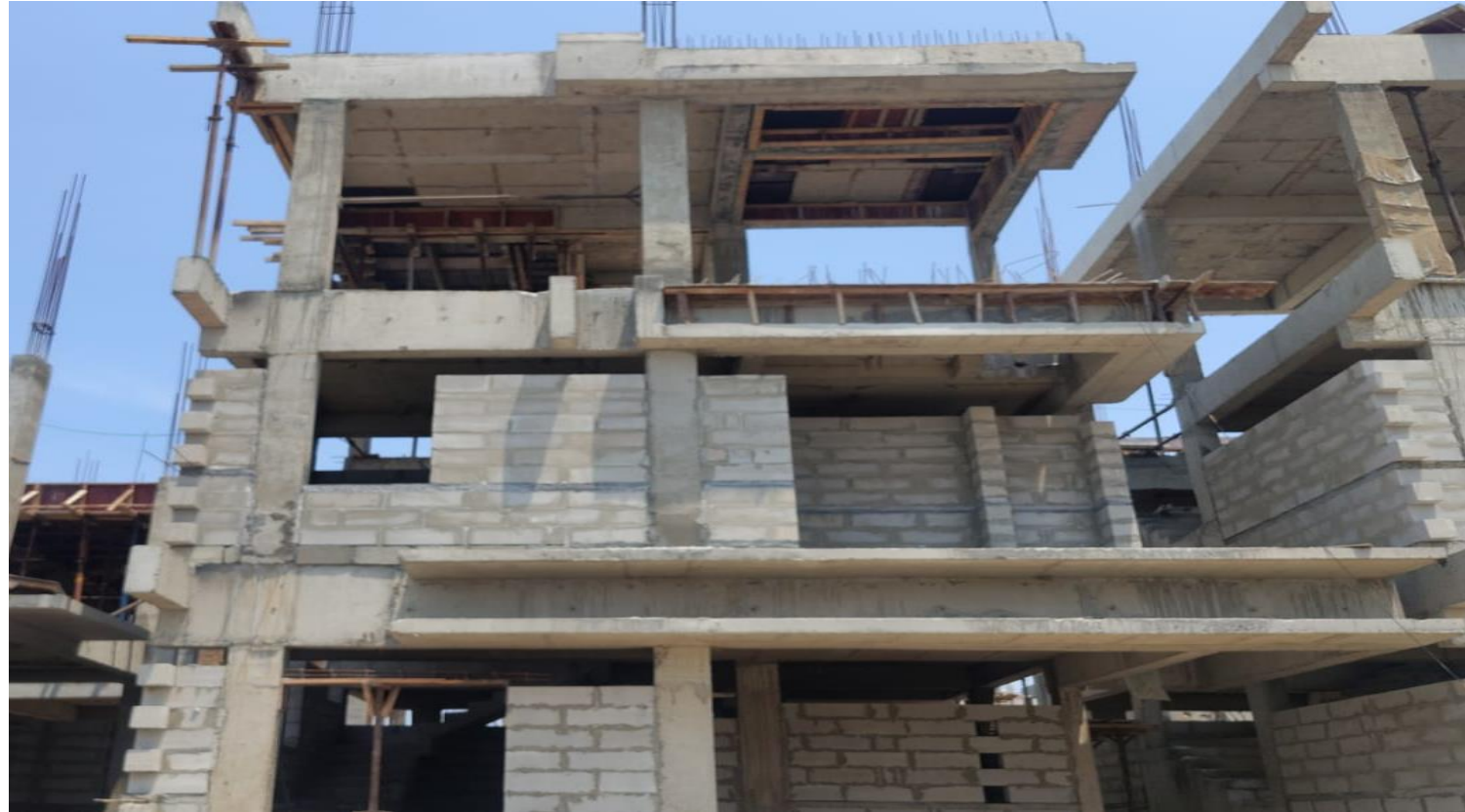
Villa No 44 –FF Block Work In Progress
