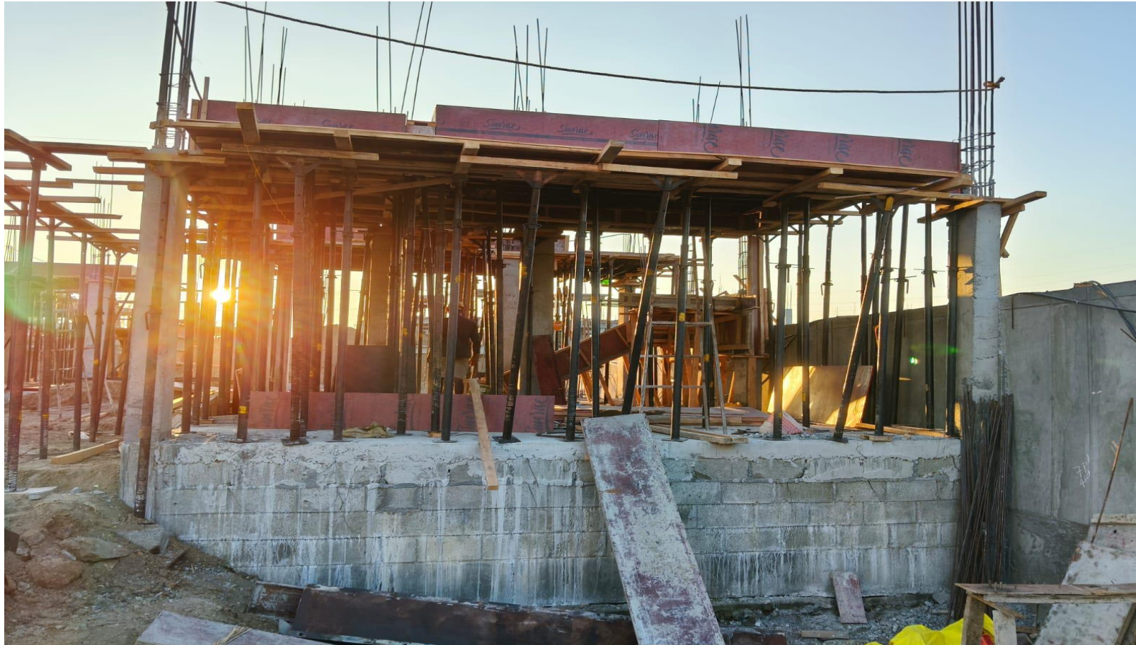
Villa No 120–GF Roof Slab Shuttering Work In Progress
