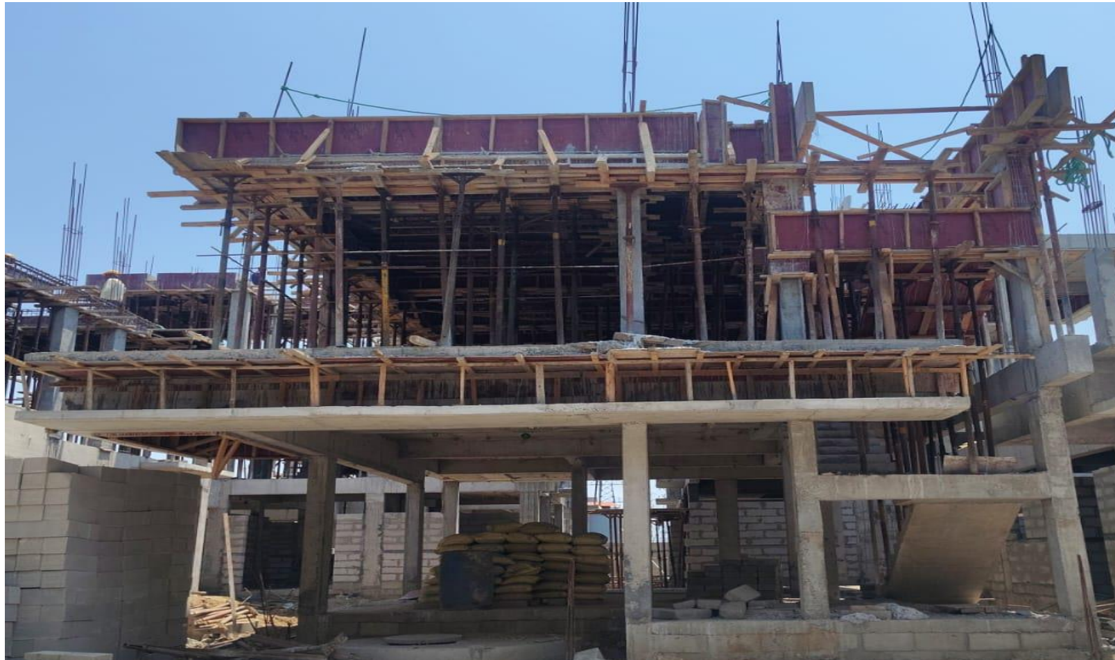
Villa No 42 –FF Roof Slab Concrete Pouring Completed
