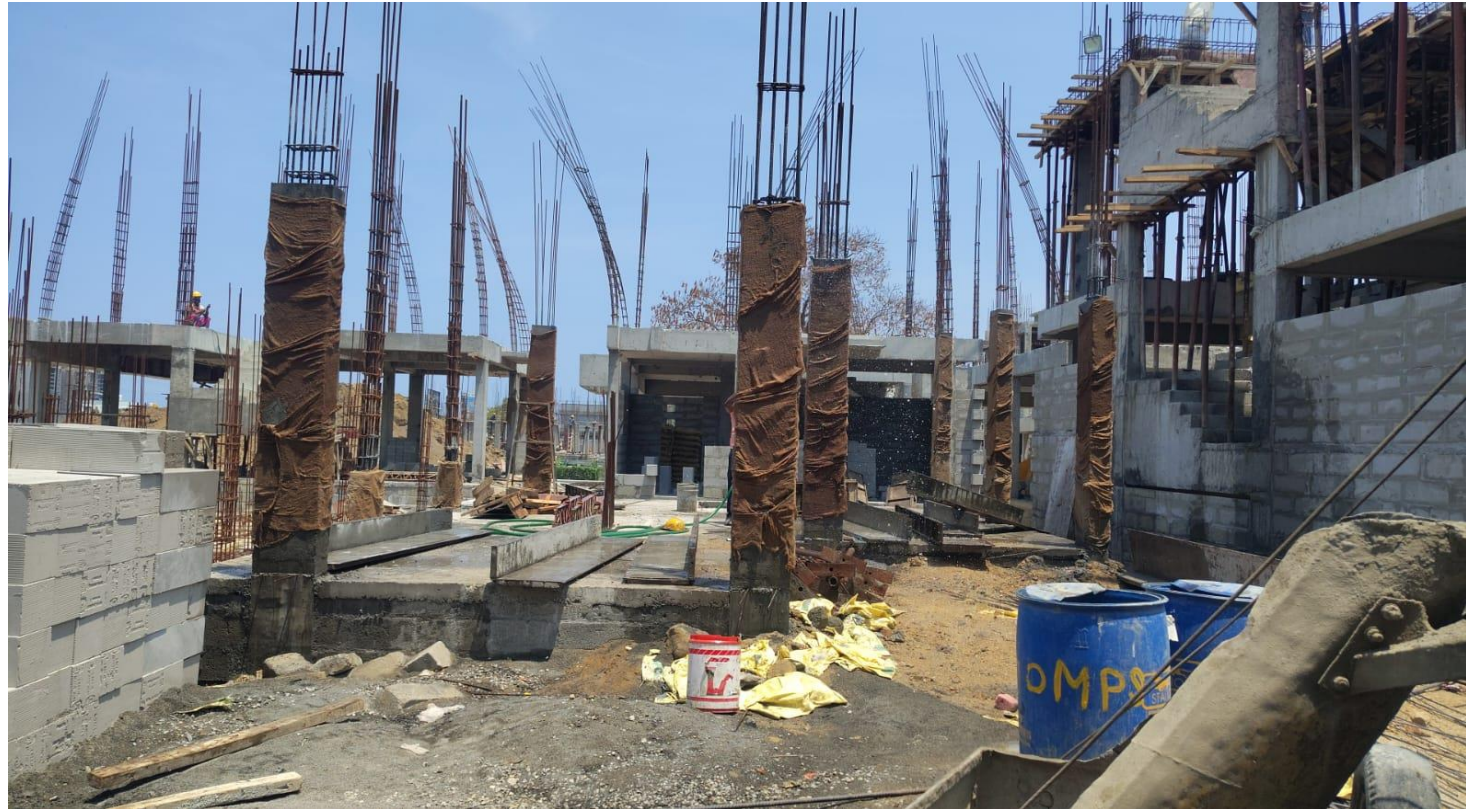
Villa No 36–GF Column Concrete work Completed
