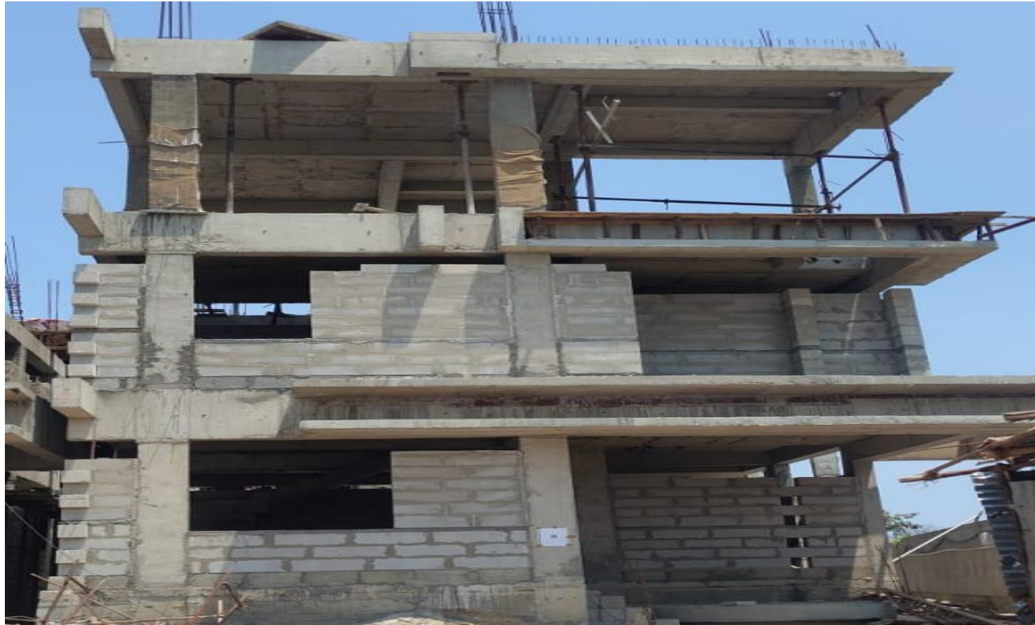
Villa No 45–FF Block Work In Progress
