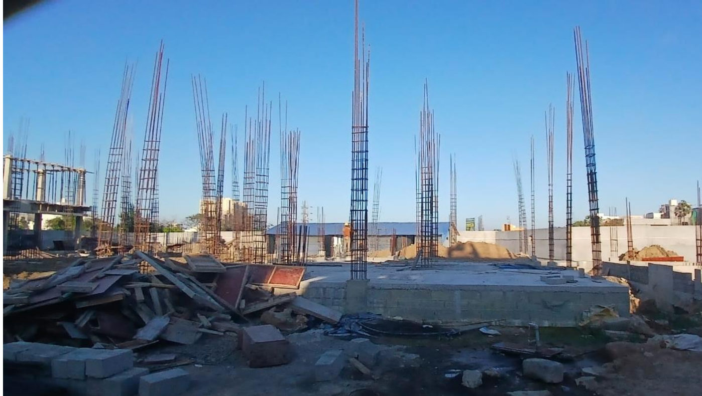
Villa No 106–GF Column Reinforcement Work Completed
