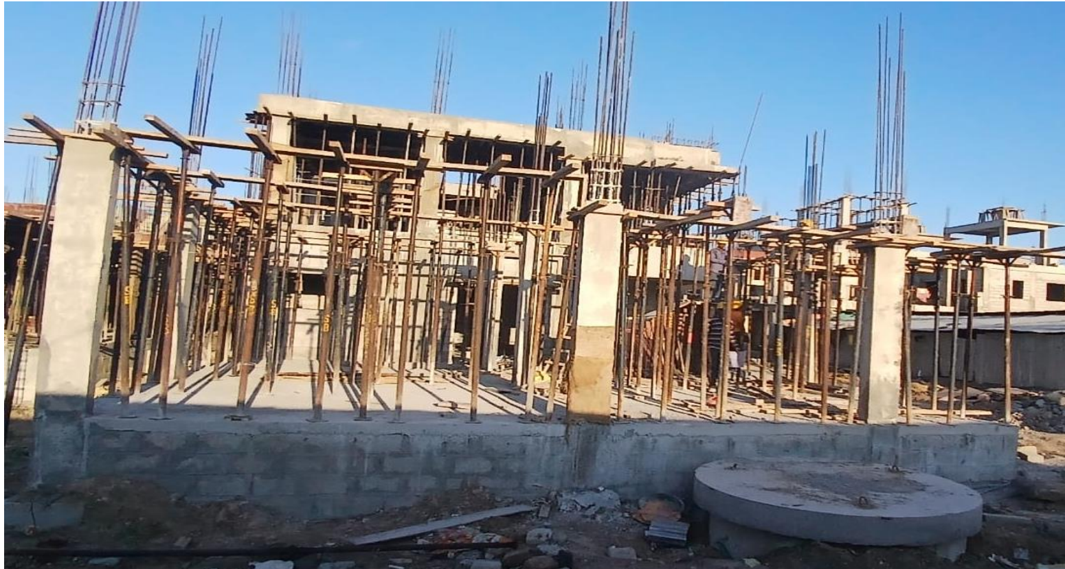
Villa No 62-GF Roof Slab Shuttering Work In Progress
