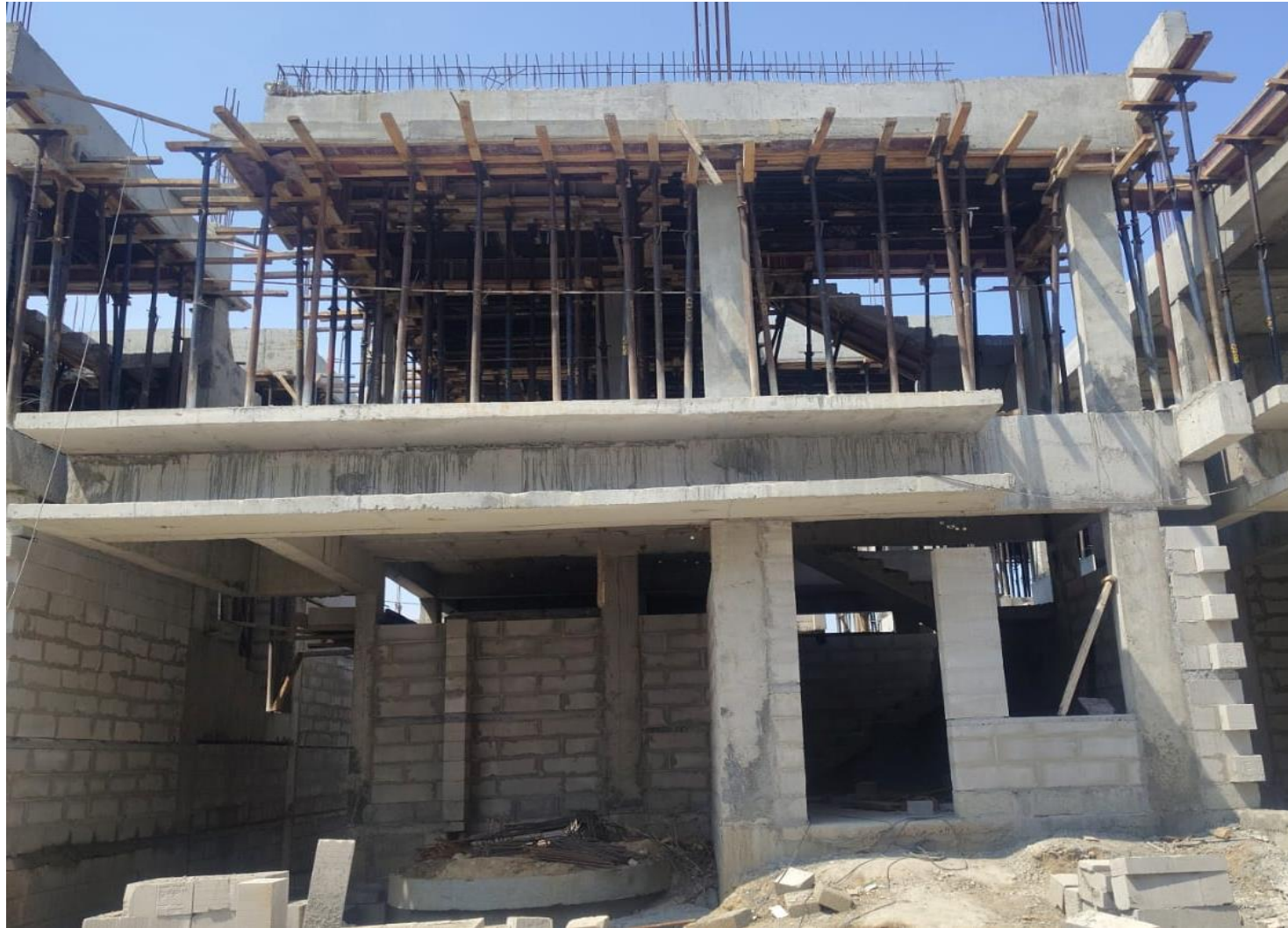
Villa No-65 FF Roof Slab Concrete Pouring Completed
