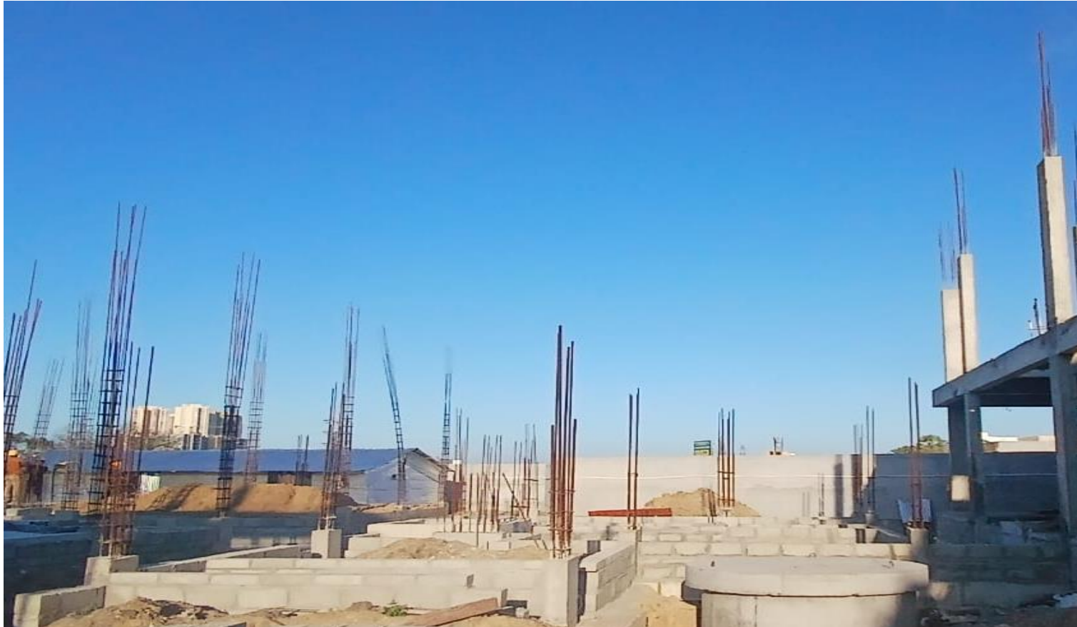
Villa No 107–Basement Block Work Completed
