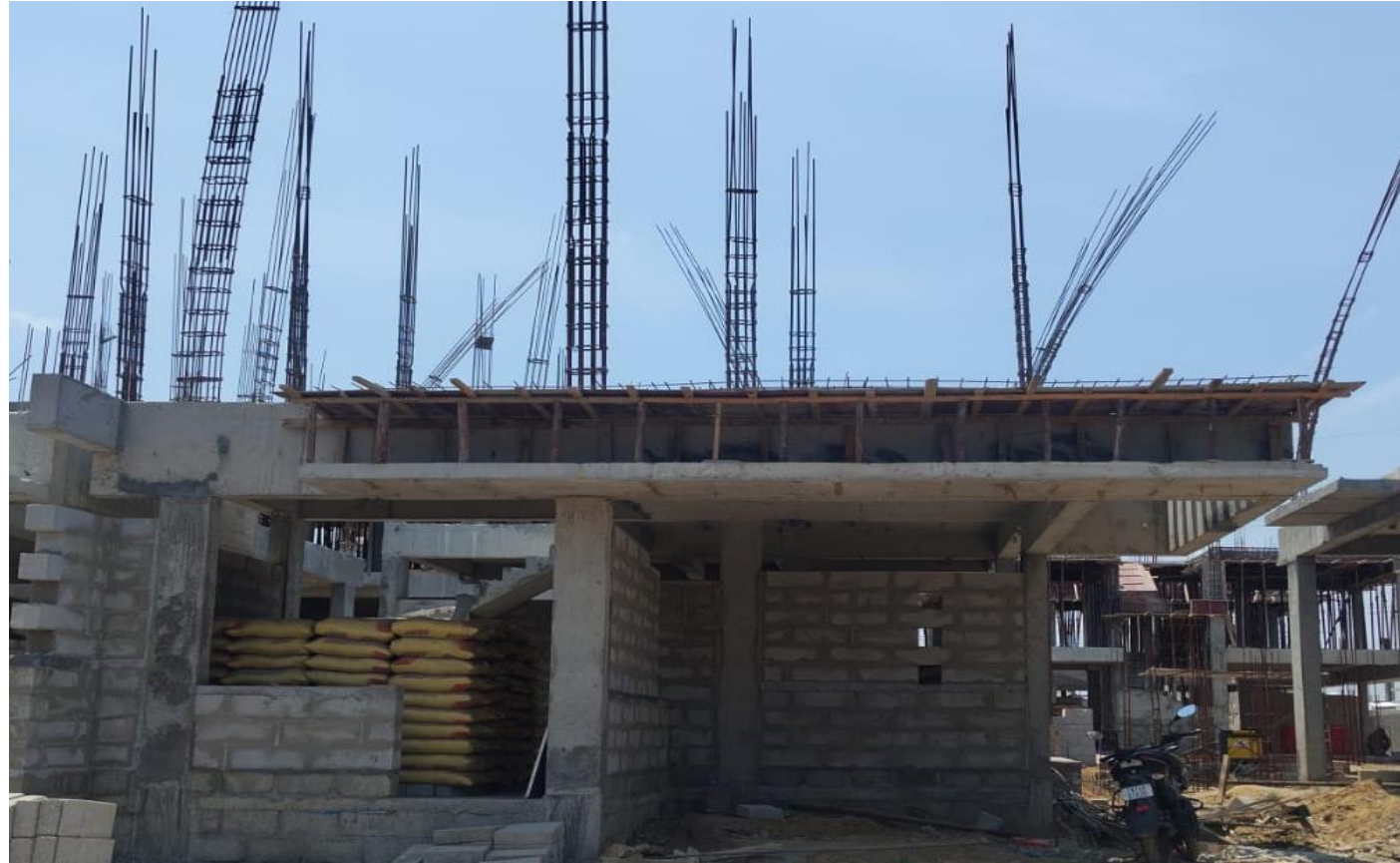
Villa No 32 –FF Column Reinforcement Work In Progress
