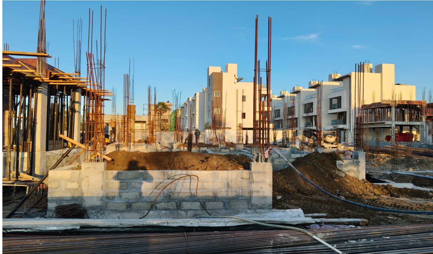
Villa No 115–Basement Block Work Completed
