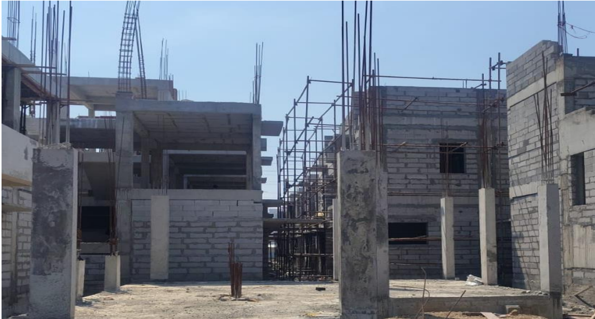
Villa No 72 –GF Column Concrete Pouring Completed
