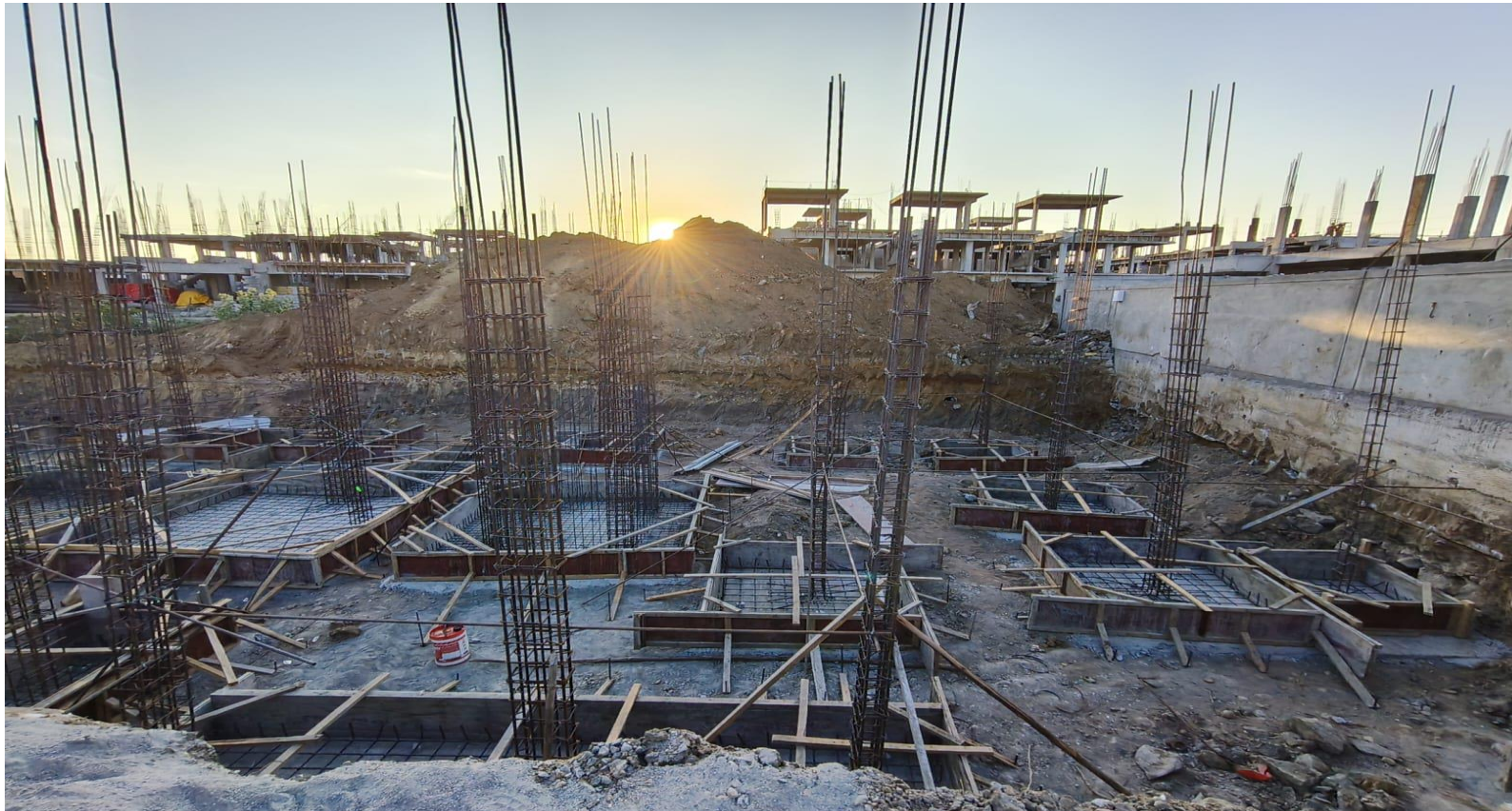
Villa No 112–Footing Shuttering Work In Progress
