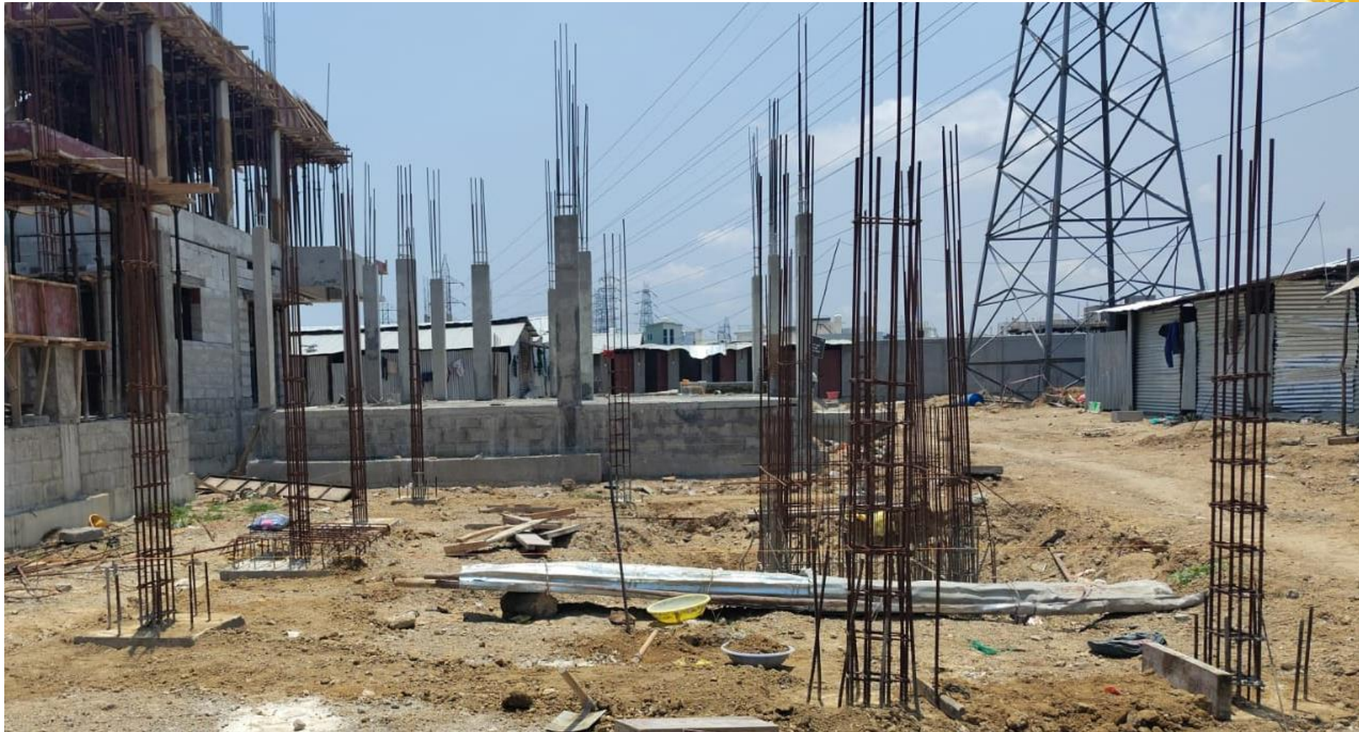
Villa No 82 – Pile Cap Concrete work Completed
