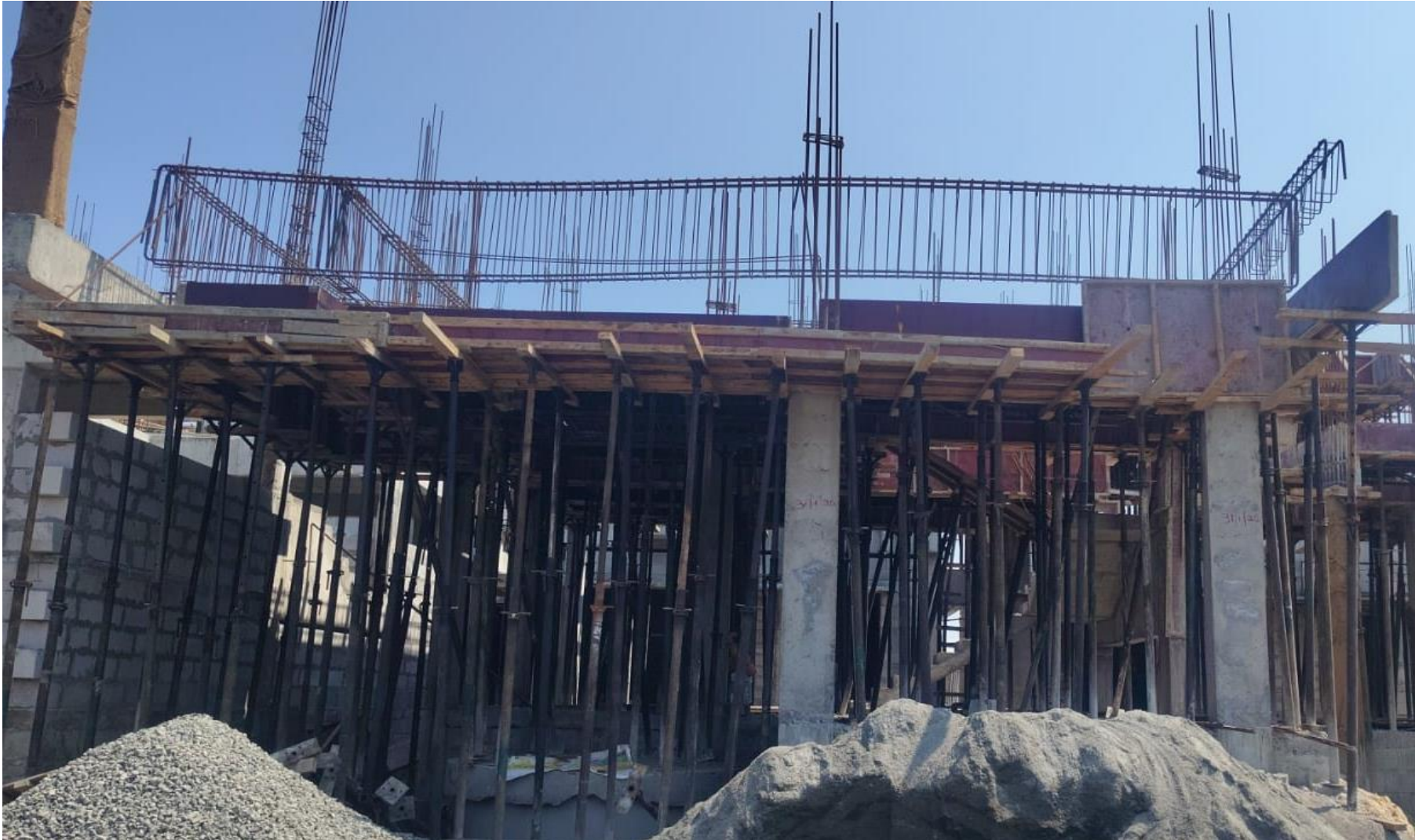
Villa No 80 –GF Roof Slab Reinforcement Work In Progress
