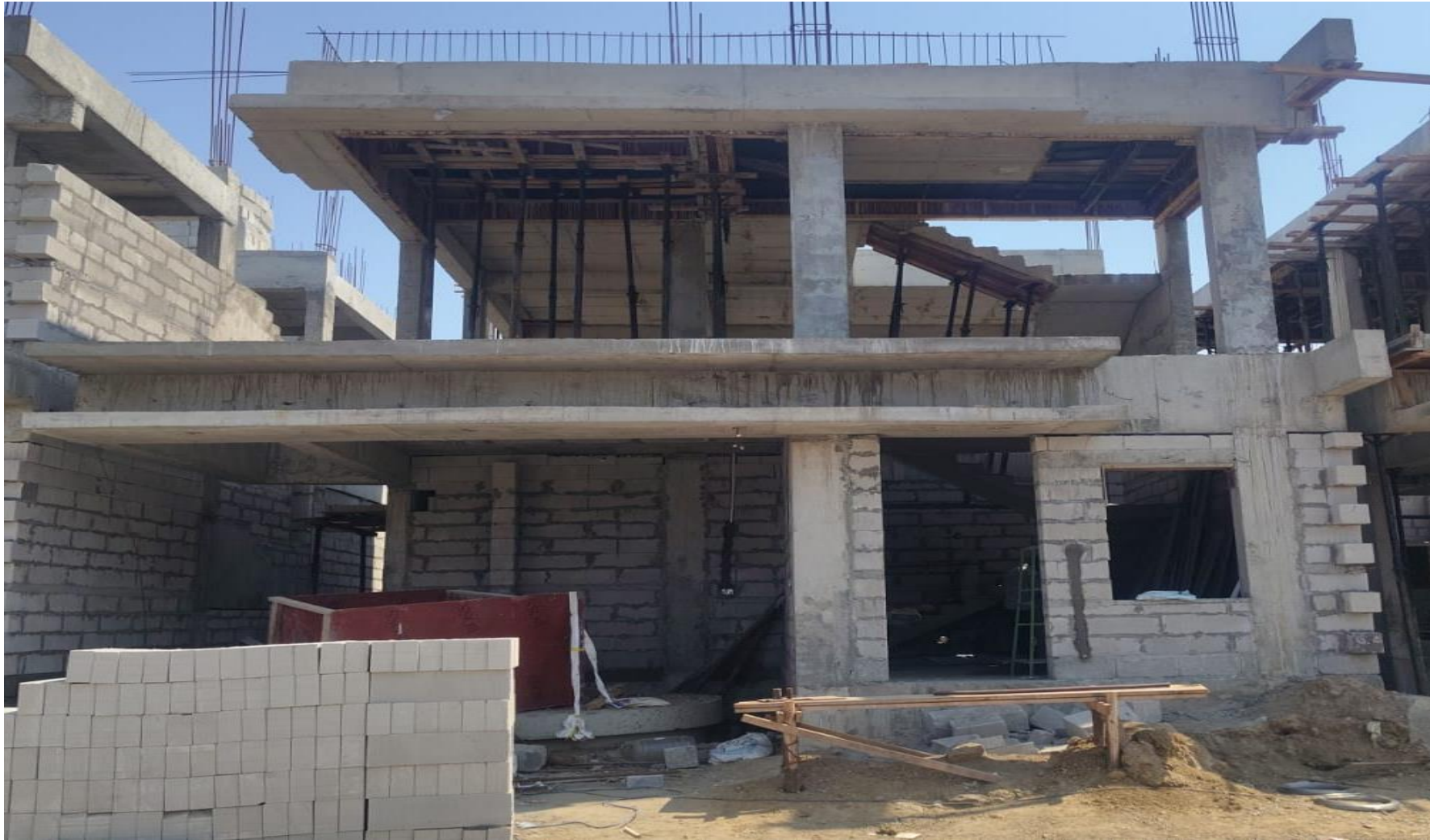
Villa No 77 –GF Block Work In Progress
