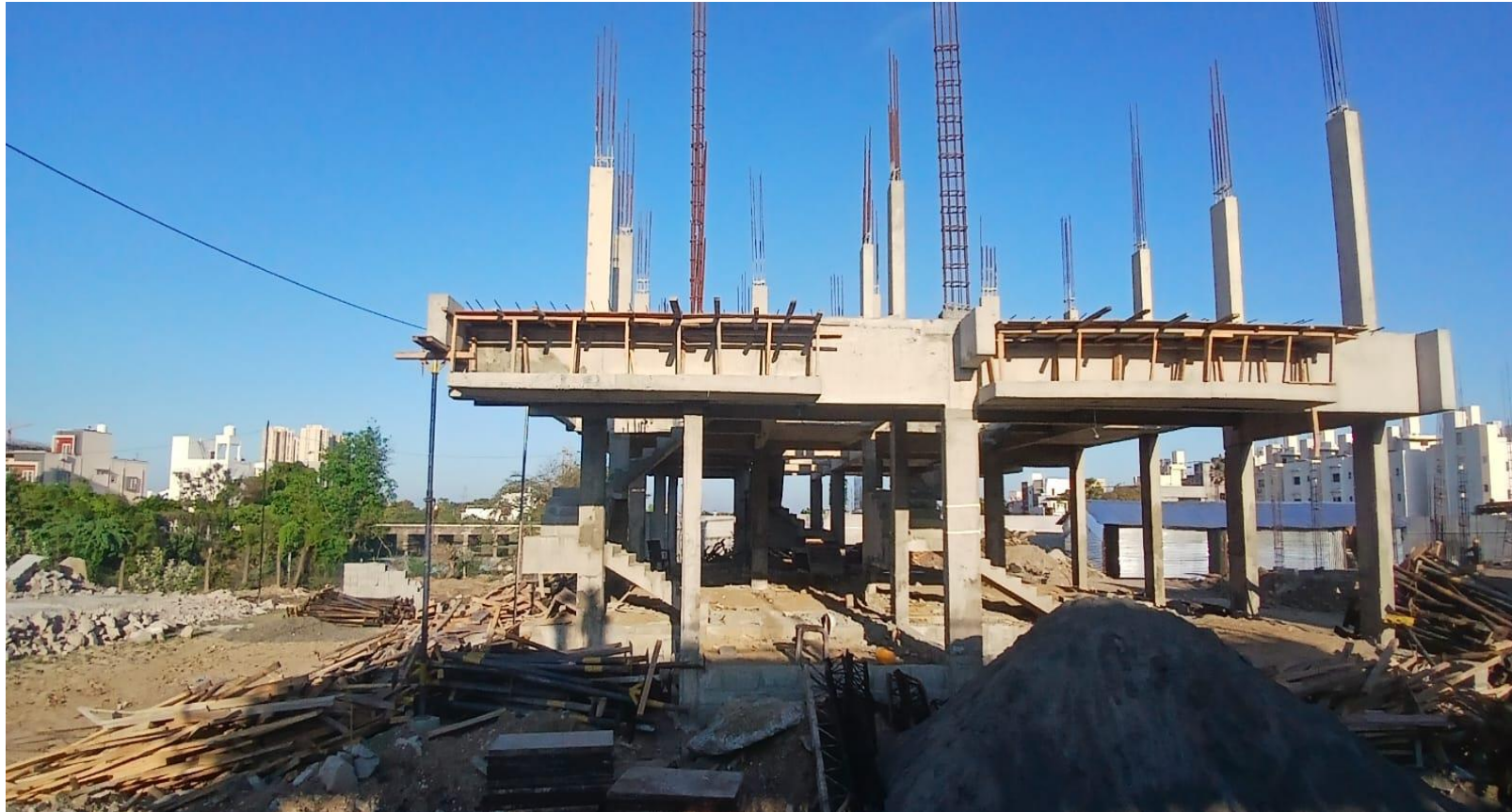
Villa No 99 to 102–FF Column Concrete Pouring Completed
