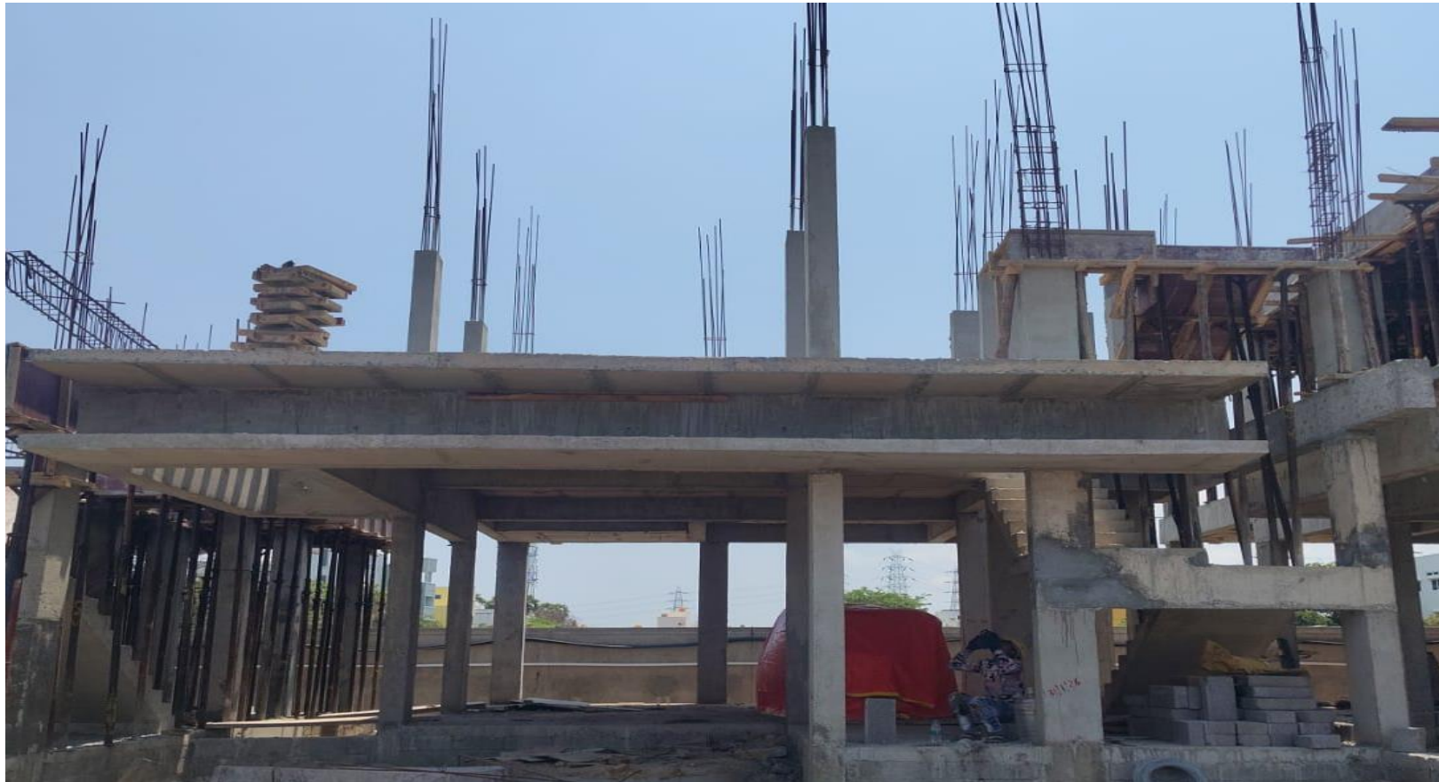
Villa No 25- FF Column Concrete Pouring Work Completed
