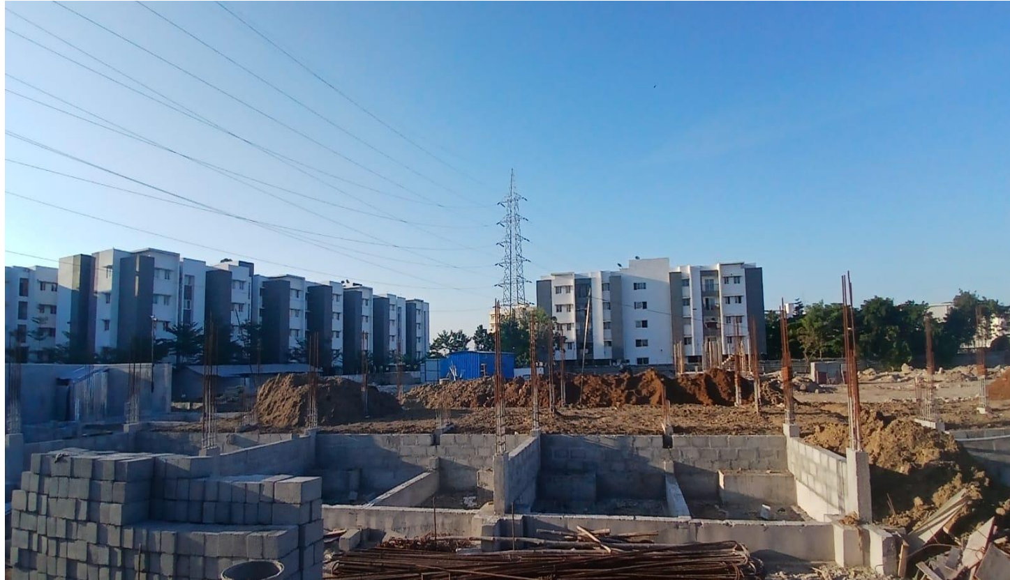
Villa No 85 & 86–Basement Block Work In Progress
