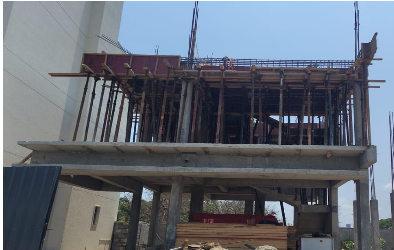
Villa No 22 –FF Roof Slab Reinforcement work In Progress
