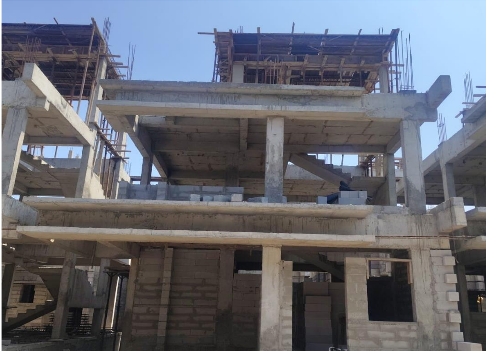
Villa No 58 –Head Room Roof Slab Concrete Pouring Completed
