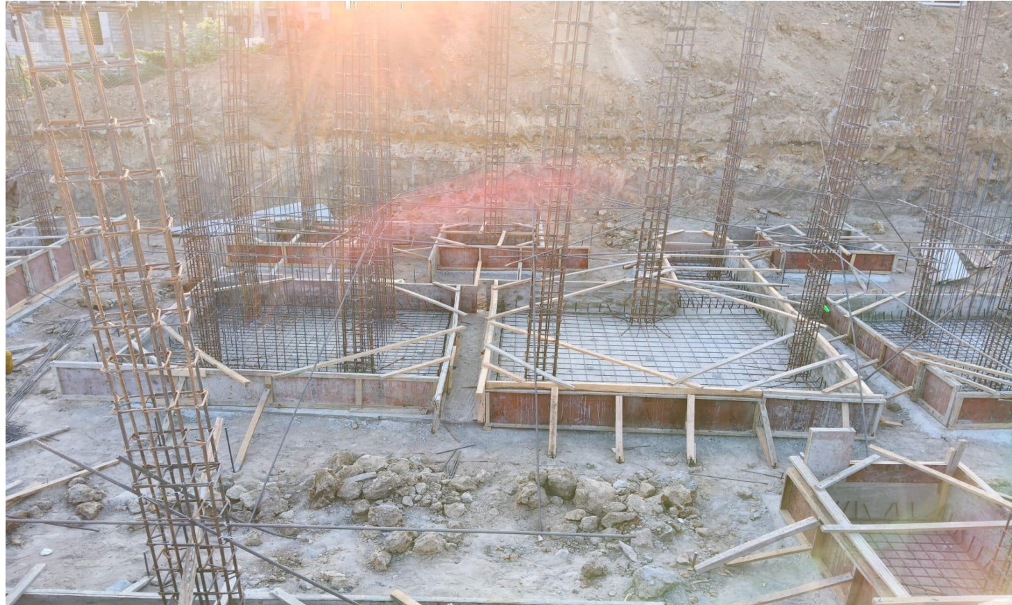
Villa No 111–Footing Shuttering Work In Progress
