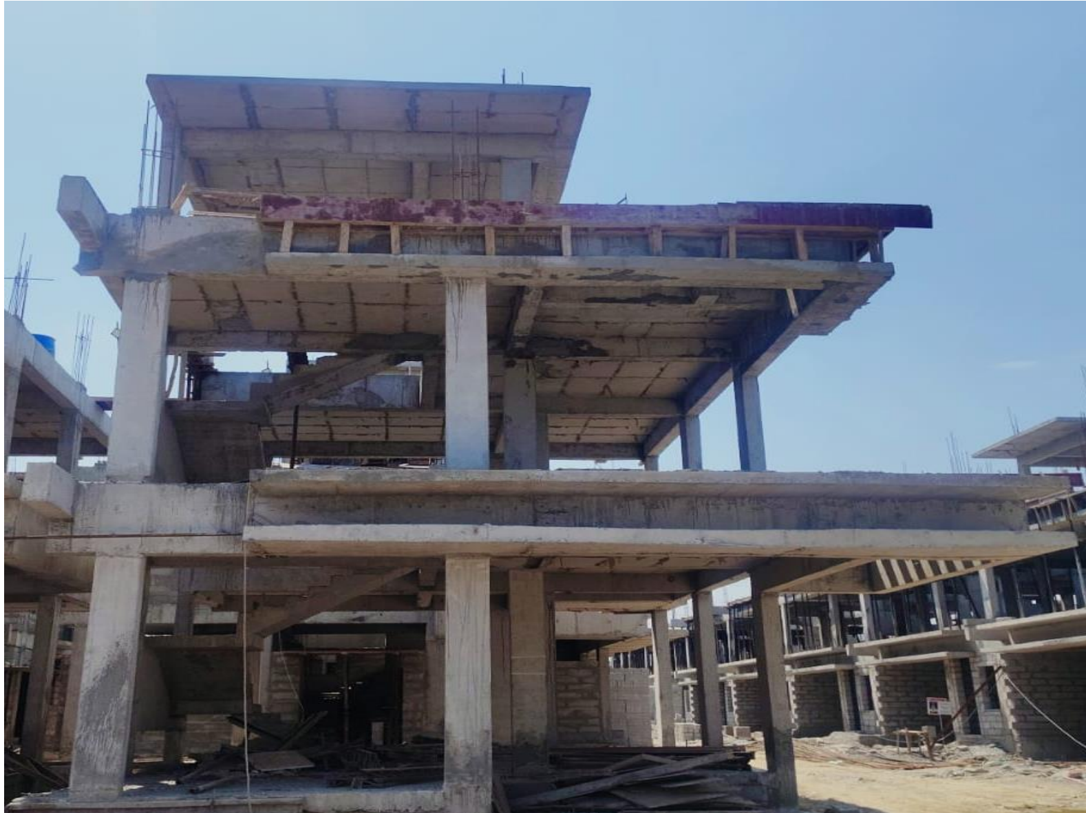
Villa No 55- Head Room Roof Slab Concrete Pouring Completed
