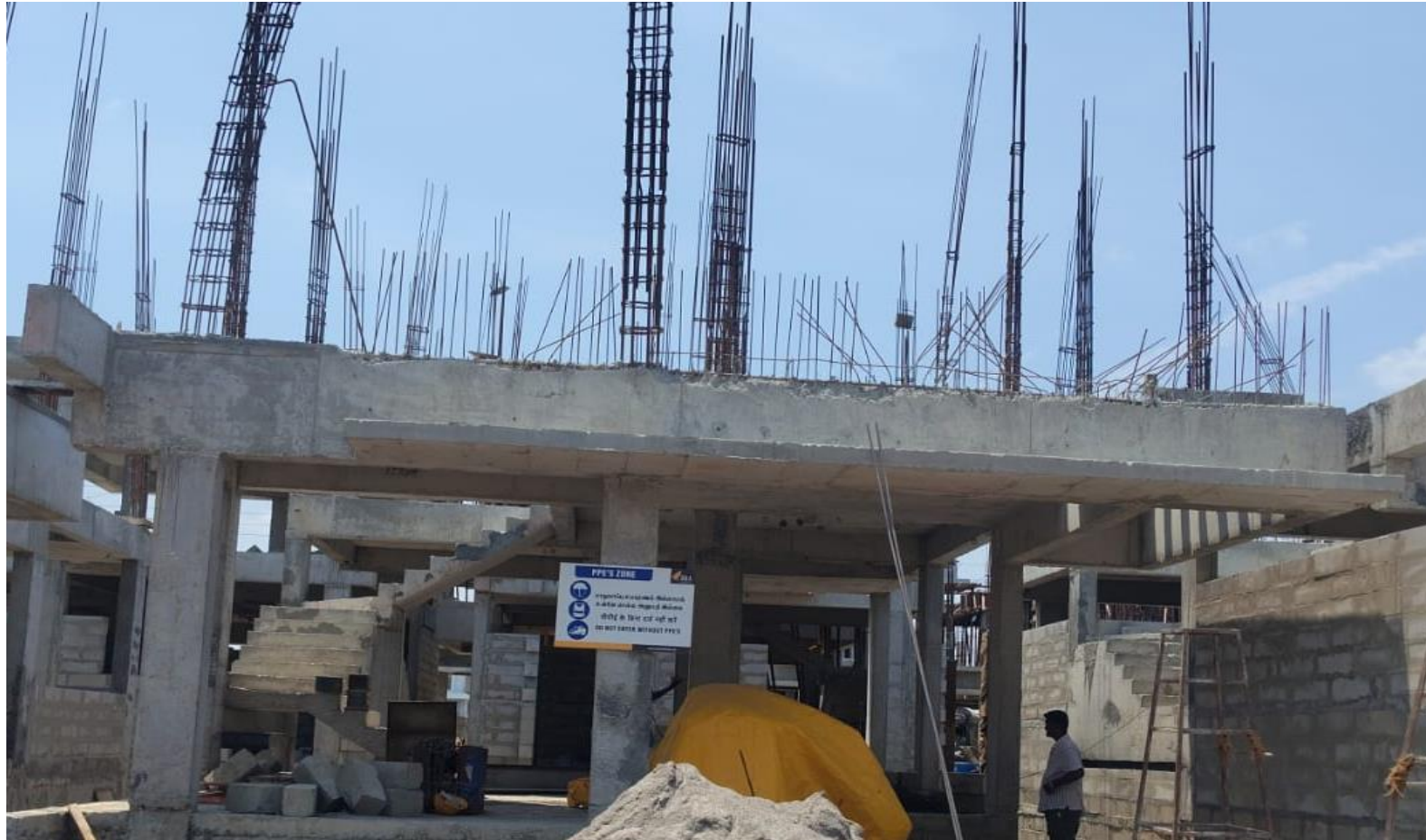
Villa No 31-FF Column Reinforcement Work In Progress
