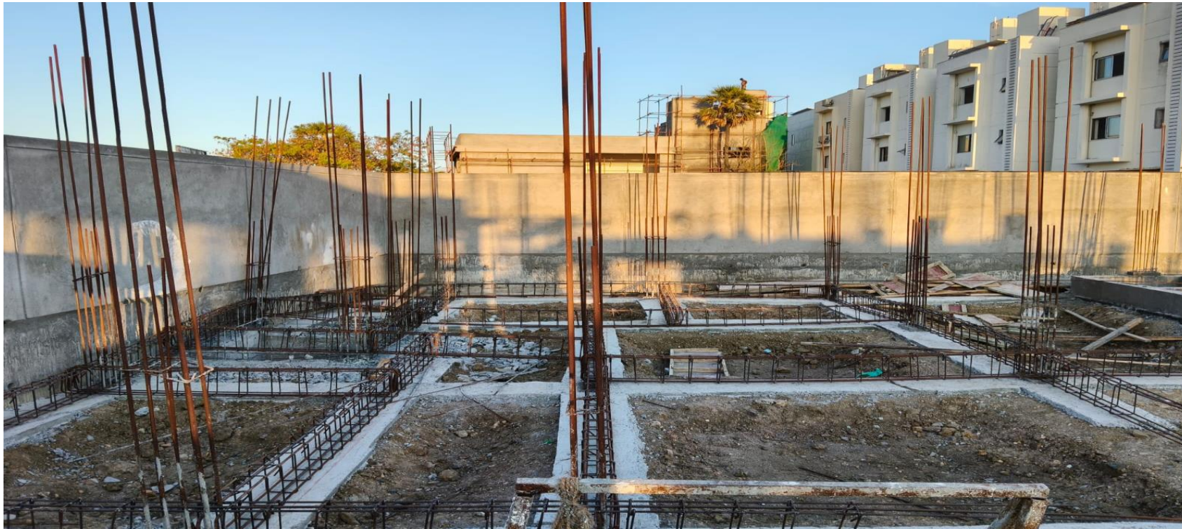
Villa No 121–Plinth Beam Reinforcement Work In Progress
