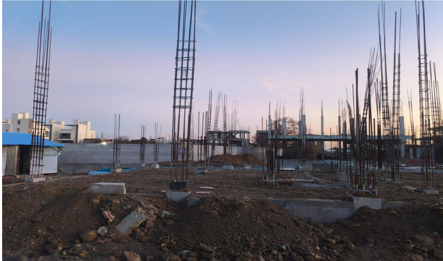
Villa No 103–Basement Back Filling Work Completed
