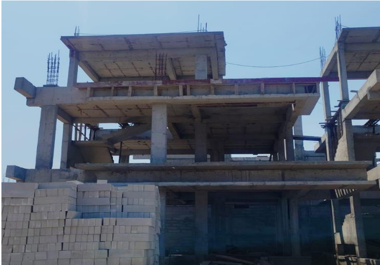
Villa No-53 Head Room Roof Slab Concrete Pouring Completed
