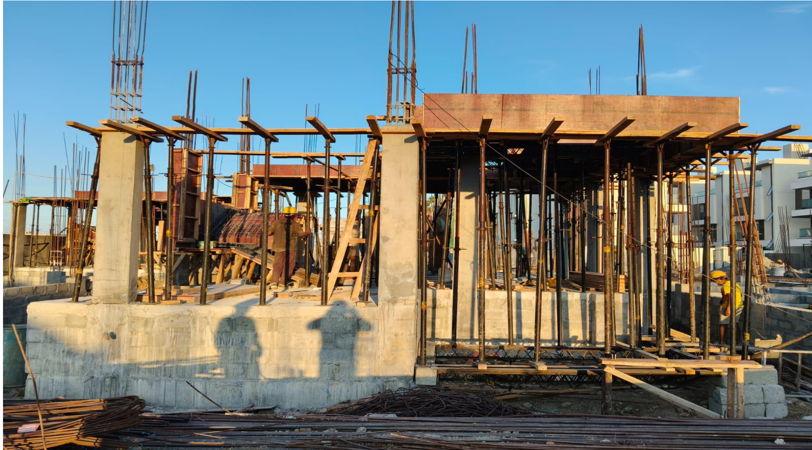
Villa No 114-GF Roof Slab Shuttering Work In Progress
