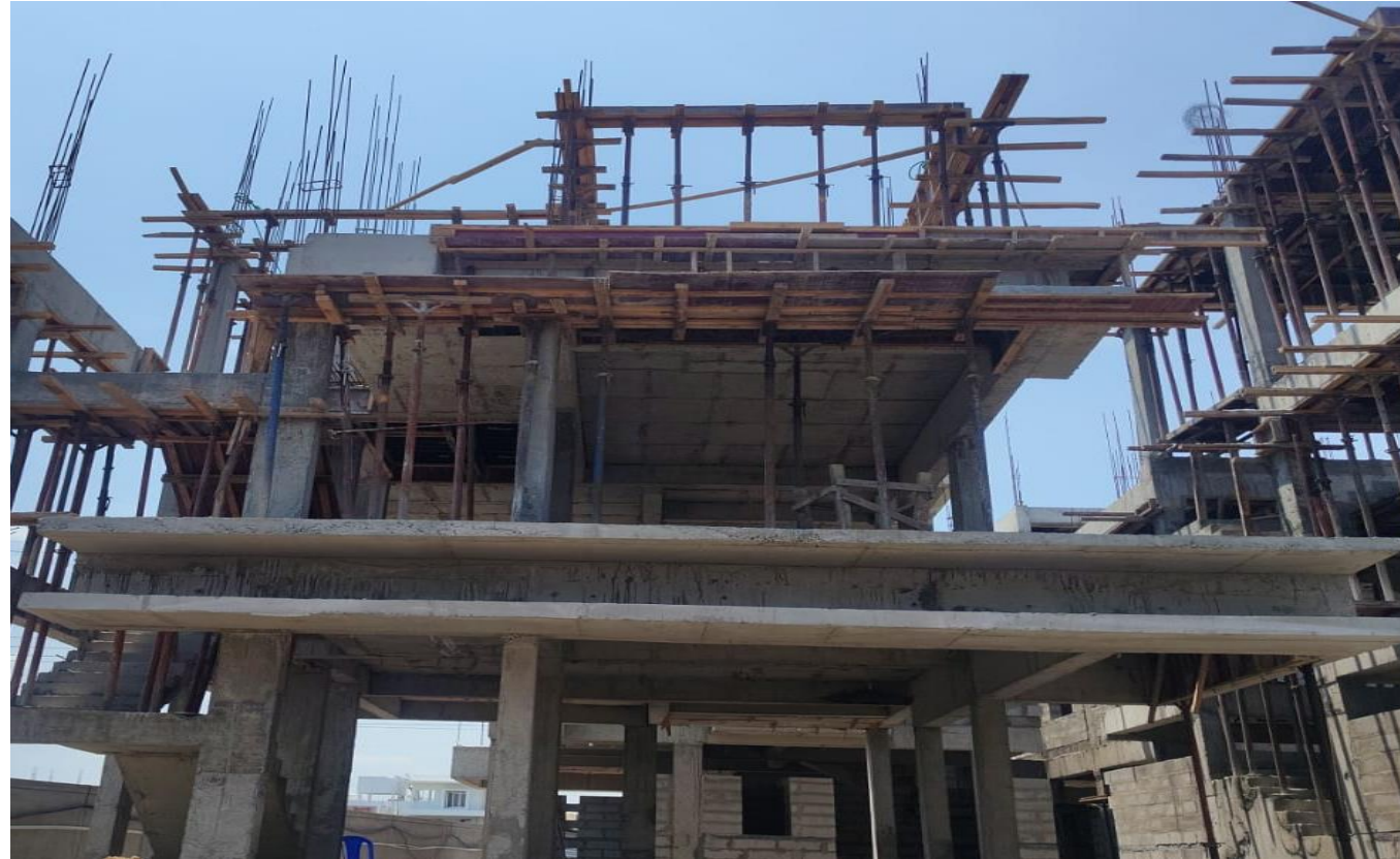
Villa No 39 –Head Room Slab Shuttering Work In Progress
