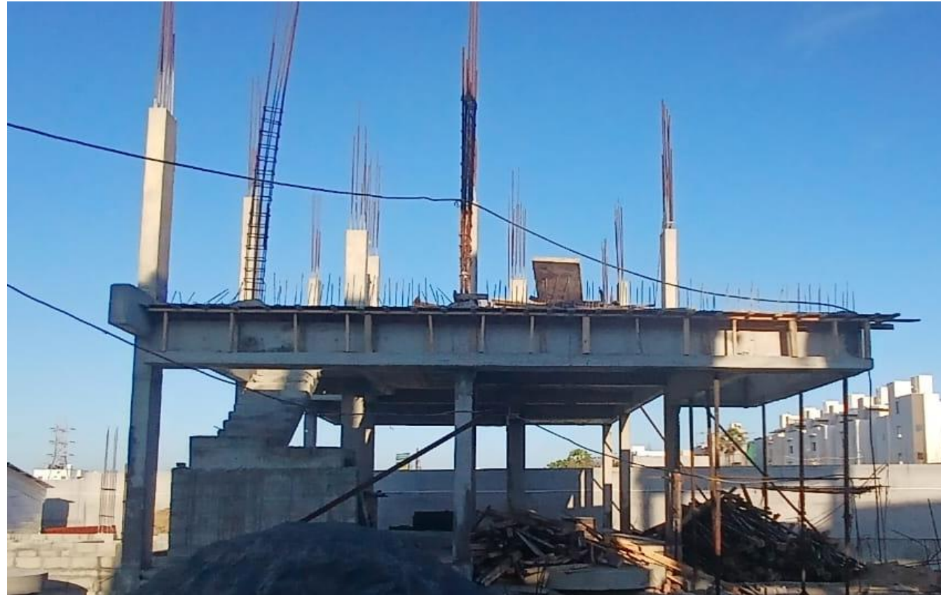
Villa No 108–FF Column Concrete Pouring Completed
