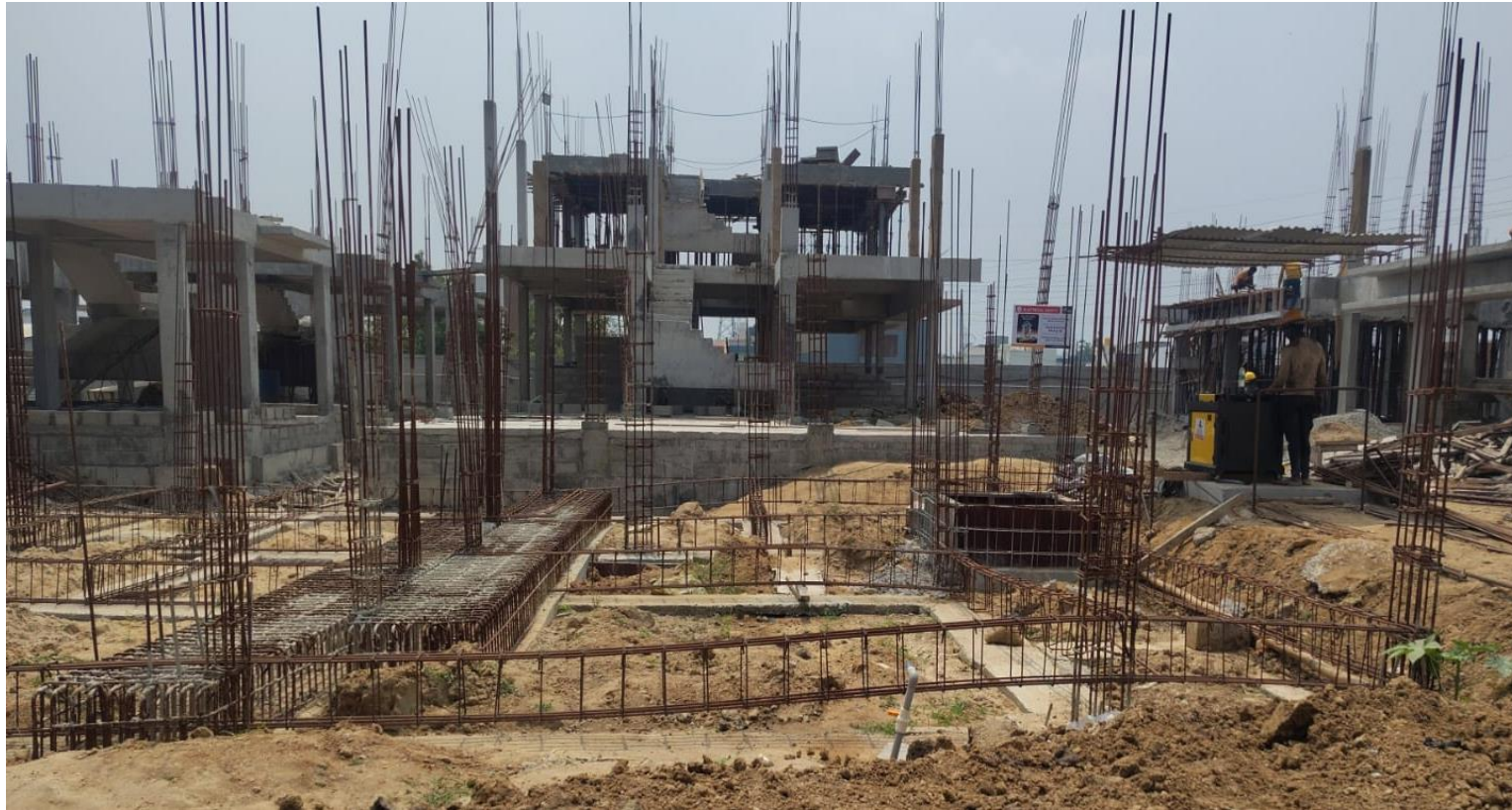
Villa No 35 –Plinth Beam Reinforcement Work In Progress
