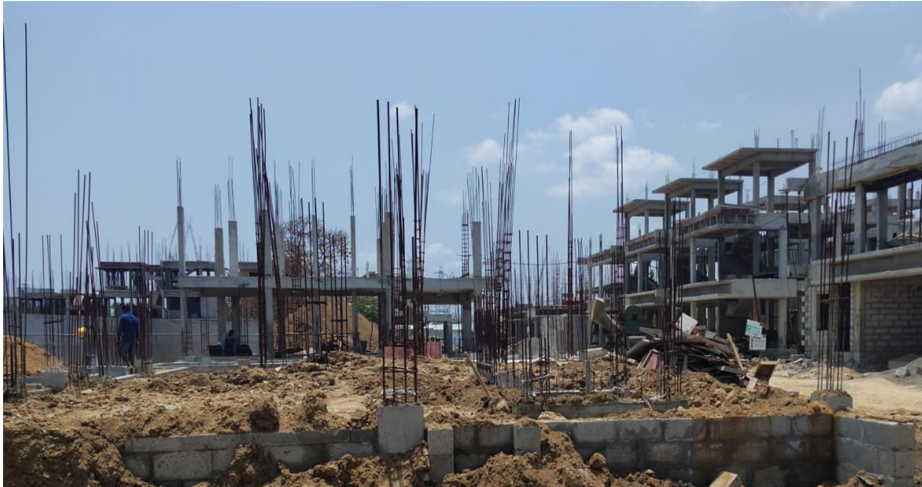
Villa No 105 – Basement Back Filling Work In Progress
