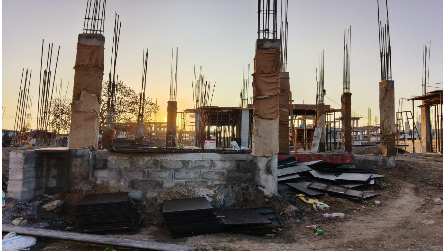
Villa No 119–GF Column Concrete Pouring Work Completed
