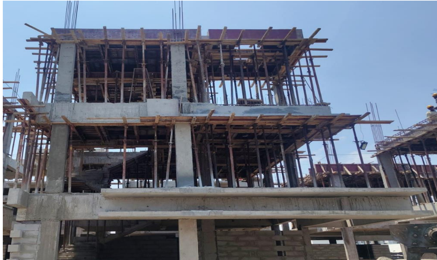
Villa No 40–Head Room Slab Shuttering Work In Progress
