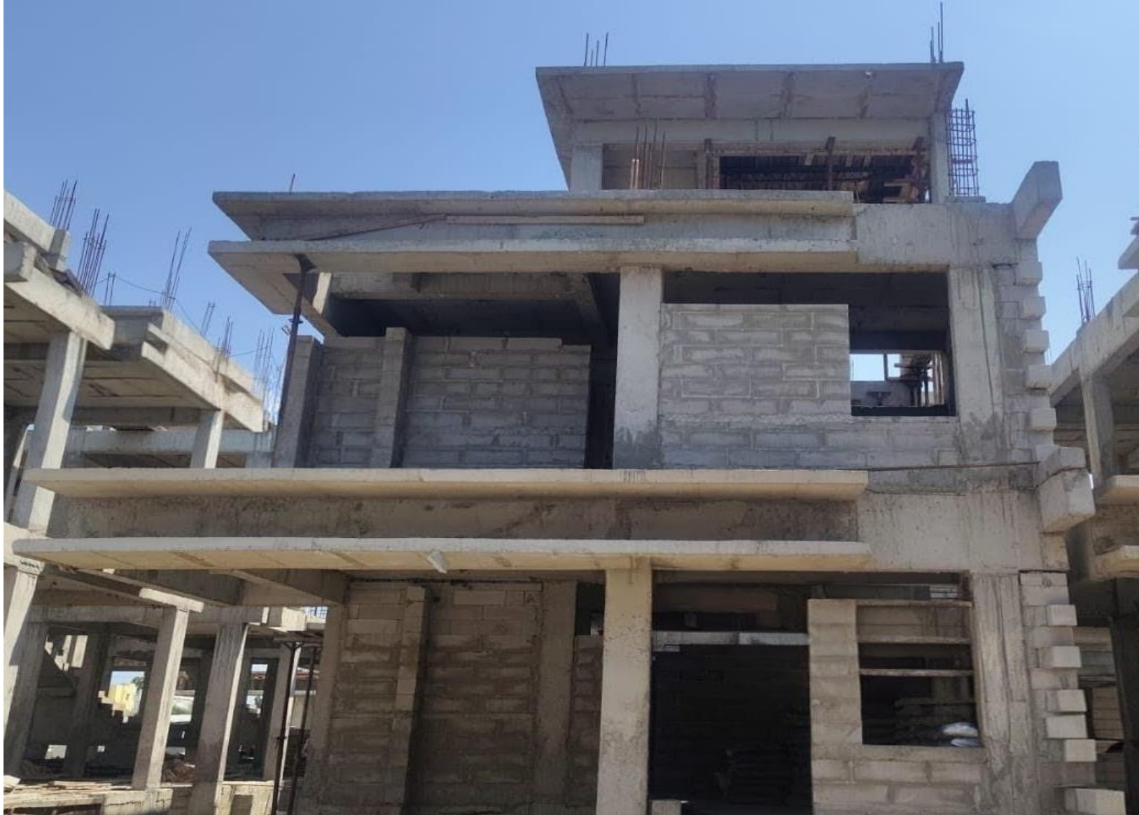
Villa No 56 – FF Block Work In Progress
