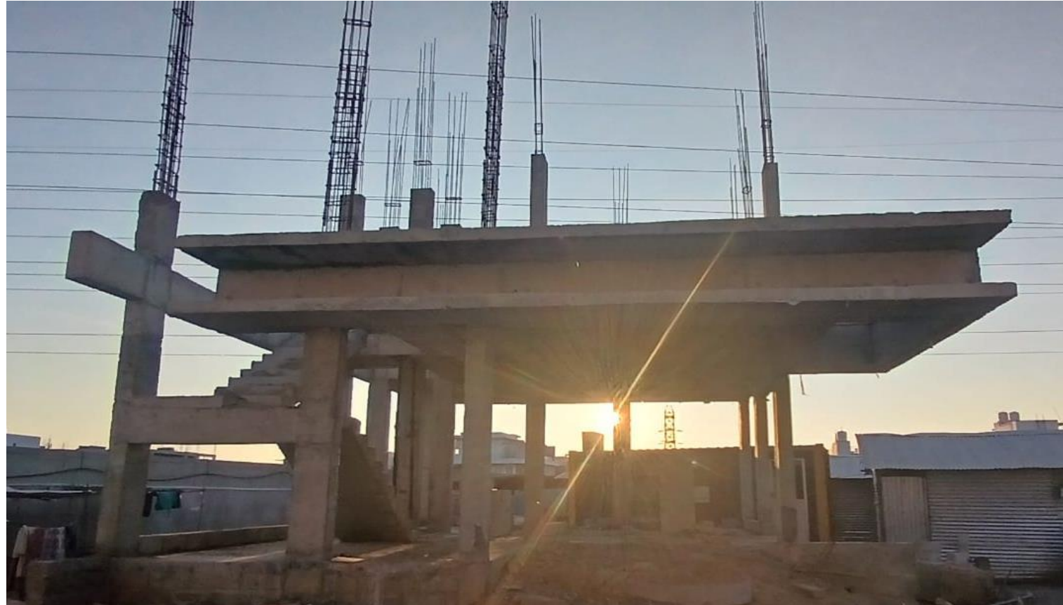
Villa No 46–FF Column Reinforcement Work Completed
