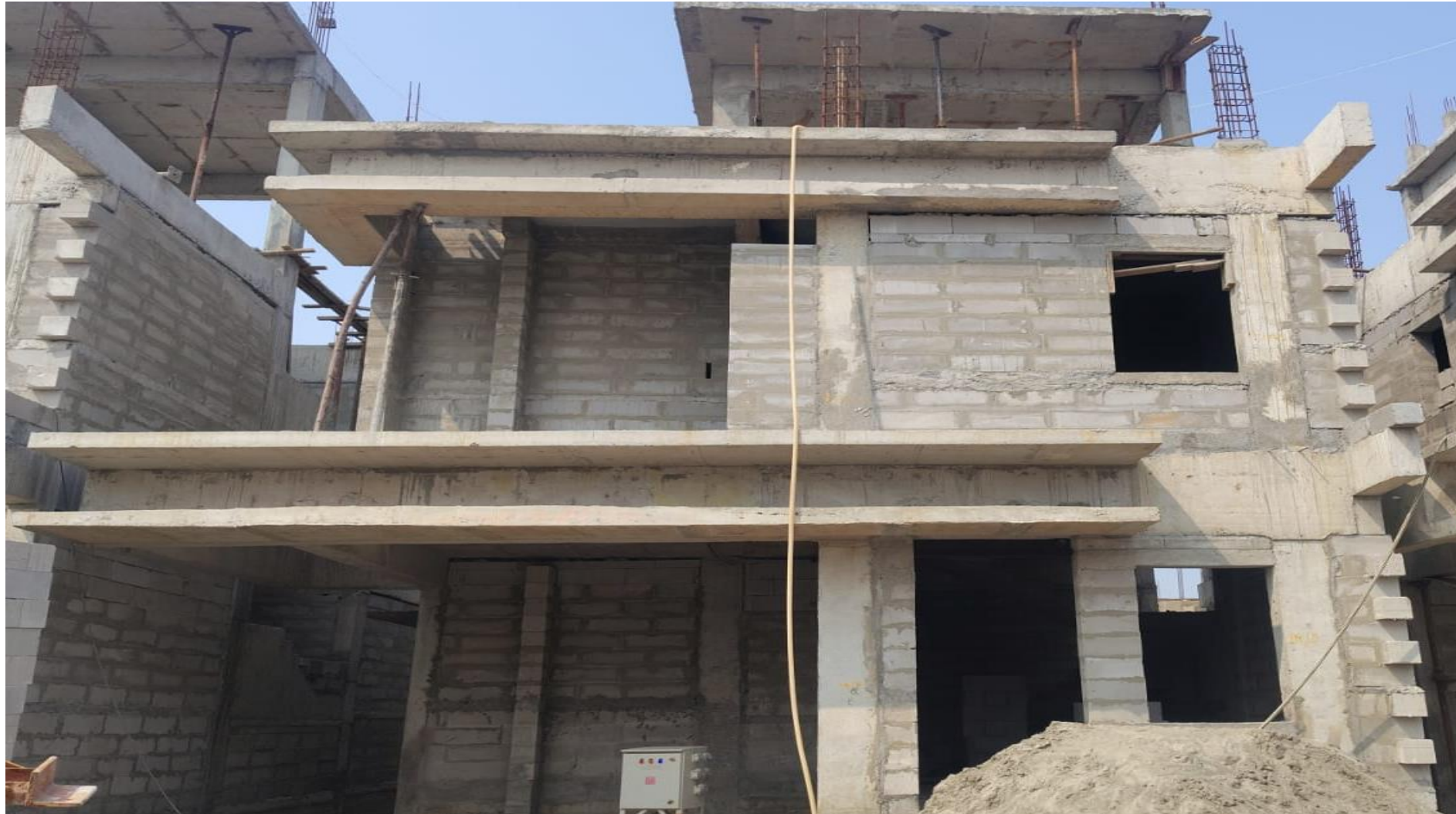
Villa No 48 –Parapet Wall Block Work In Progress
