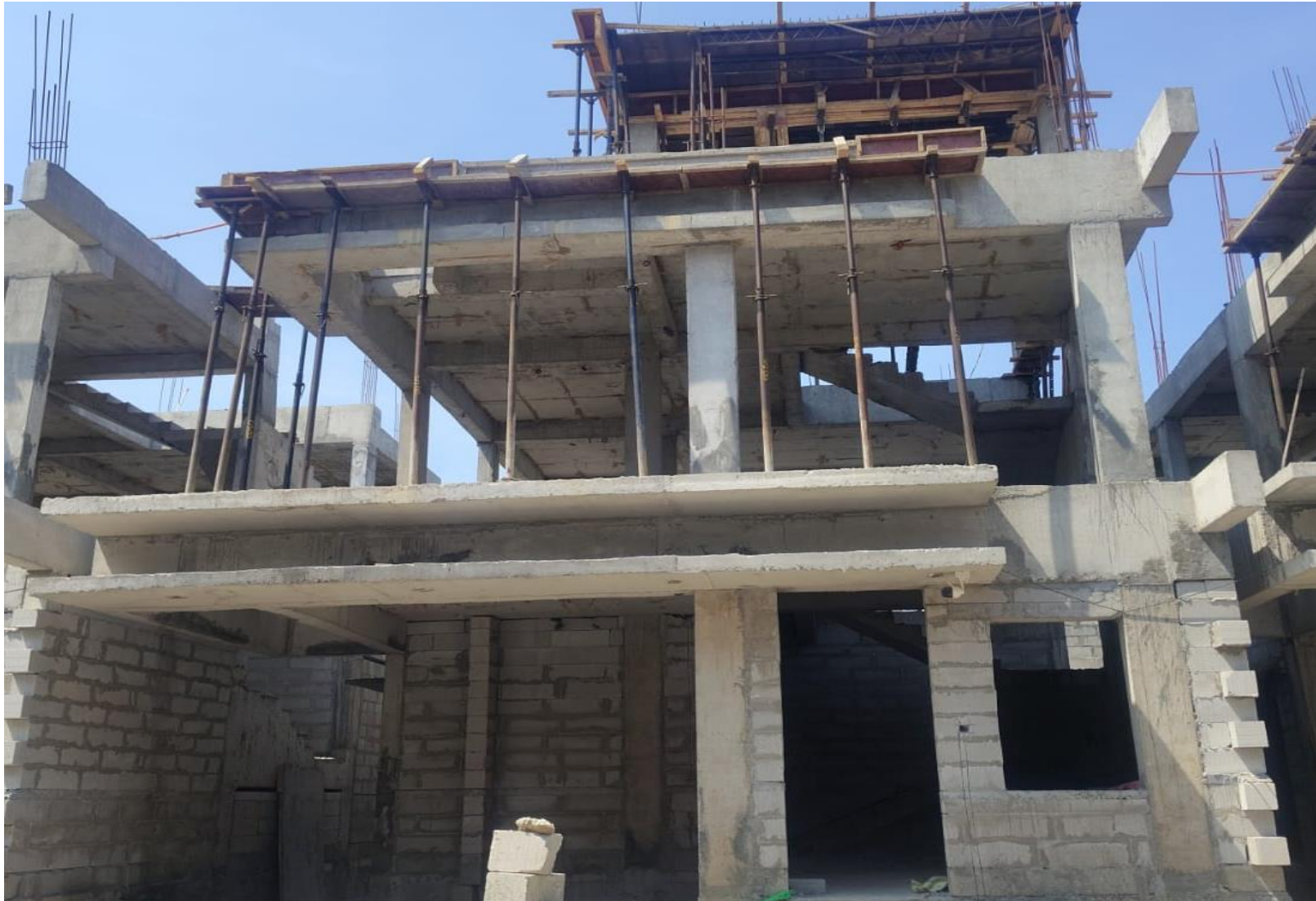
Villa No 67 –Head Room Roof Slab Concrete Pouring Completed
