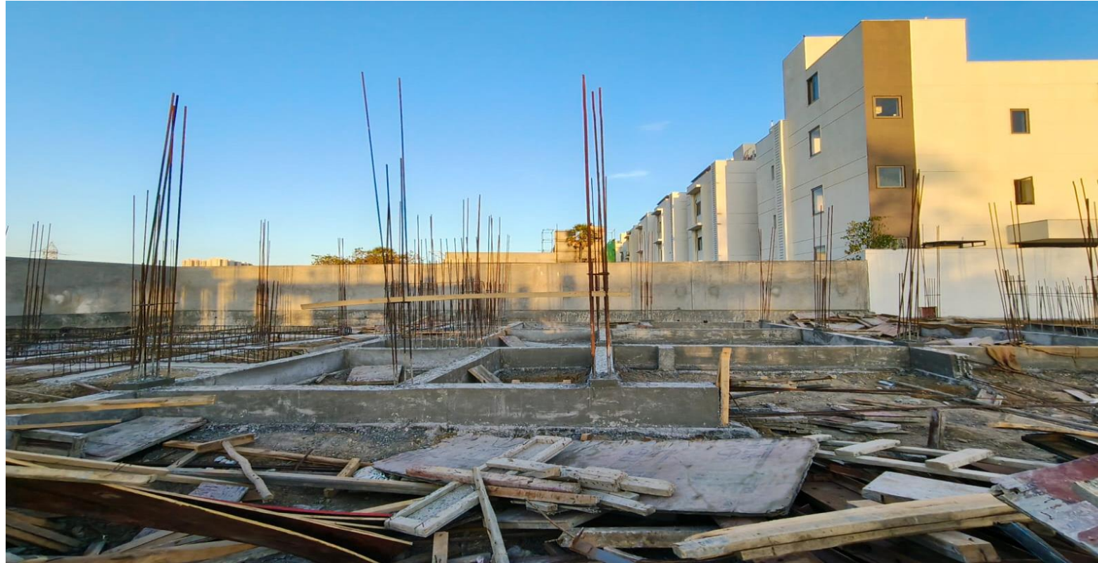
Villa No 122–Plinth Beam Concrete Pouring Completed
