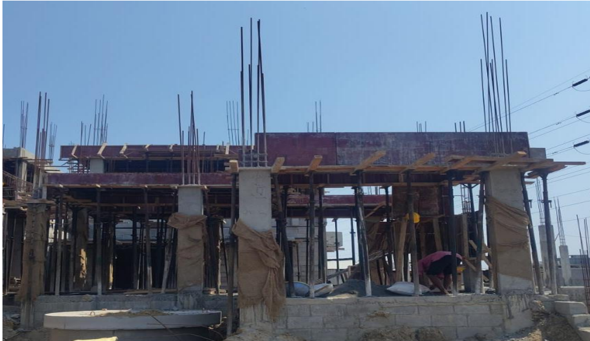
Villa No 81– GF Roof Slab Shuttering Work In Progress
