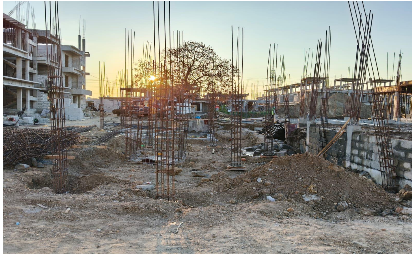
Villa No 117–Plinth Beam PCC Dressing Work In Progress
