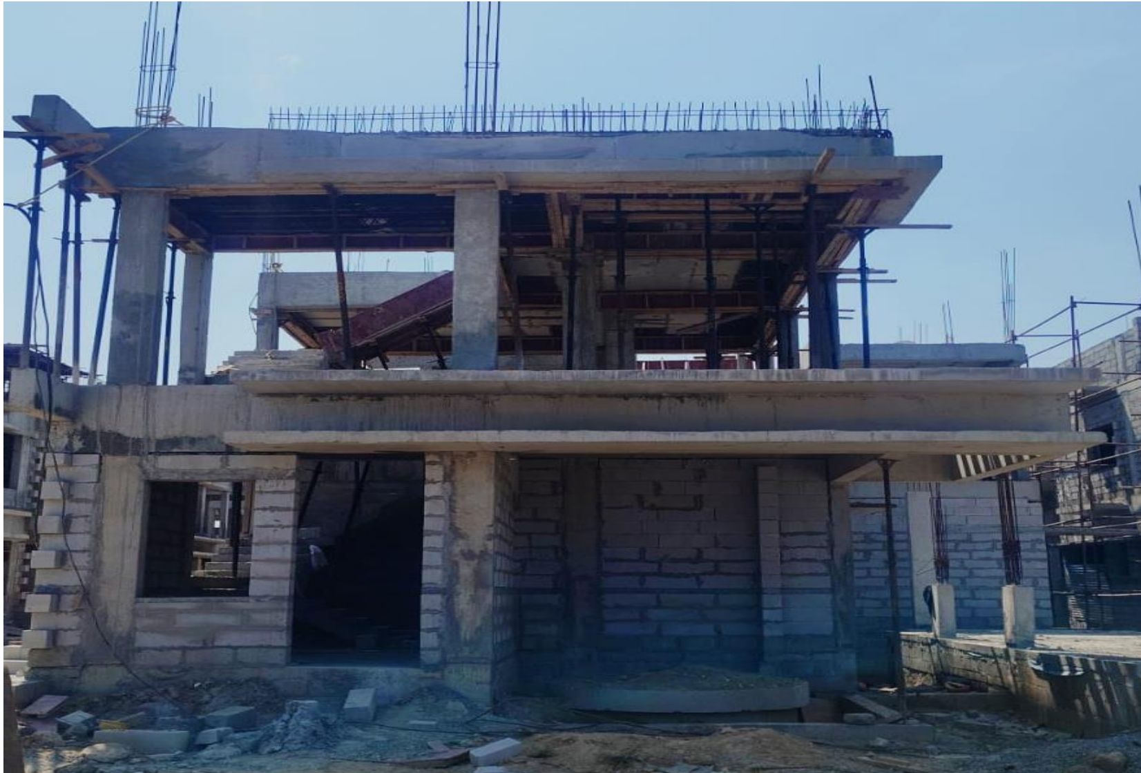
Villa No 71 – FF Roof Slab Concrete Pouring Completed
