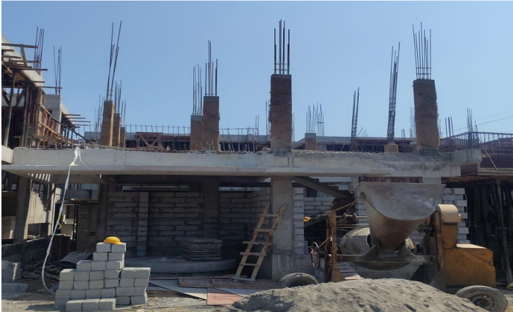
Villa No 79 –FF Column Concrete Completed
