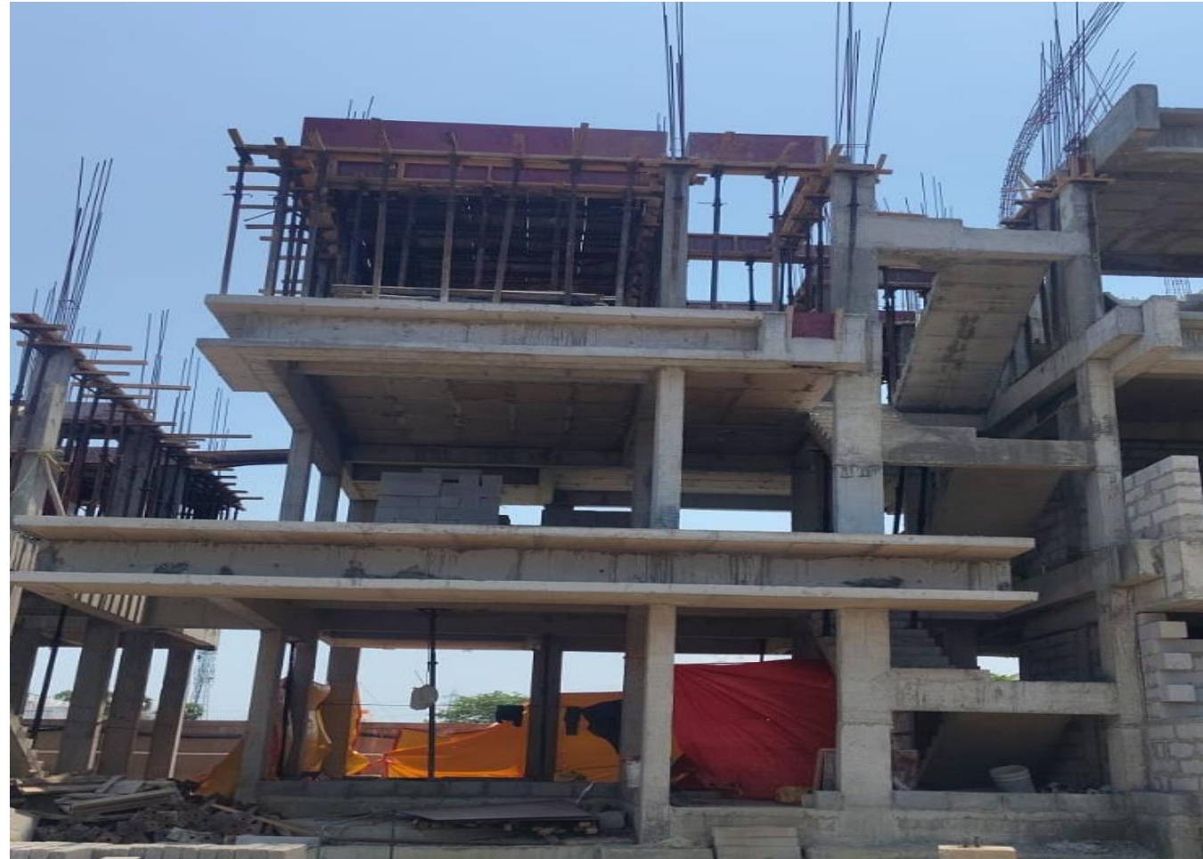
Villa No 27 –SF Roof Slab Shuttering Work In Progress
