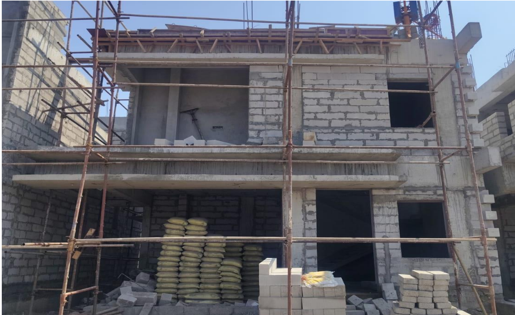
Villa No 75 –Parapet Wall Block Work In Progress
