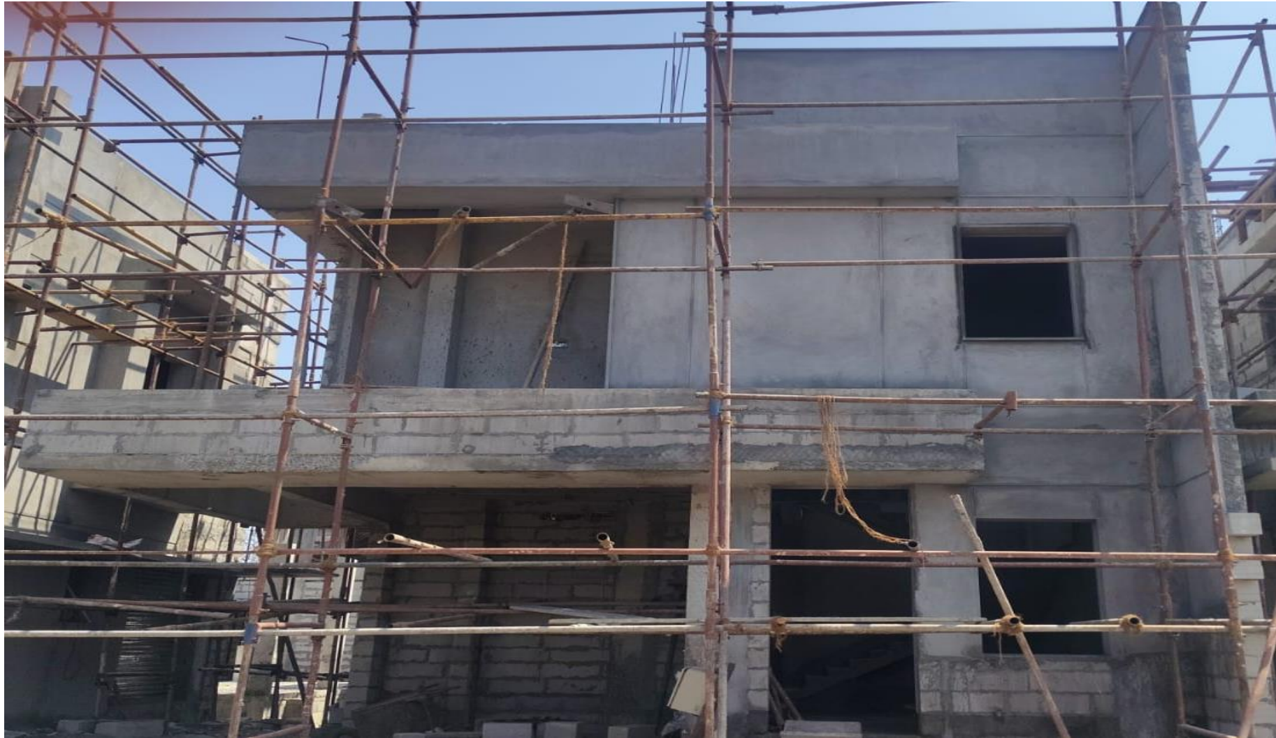
Villa No 74 – External Plastering Work In Progress
