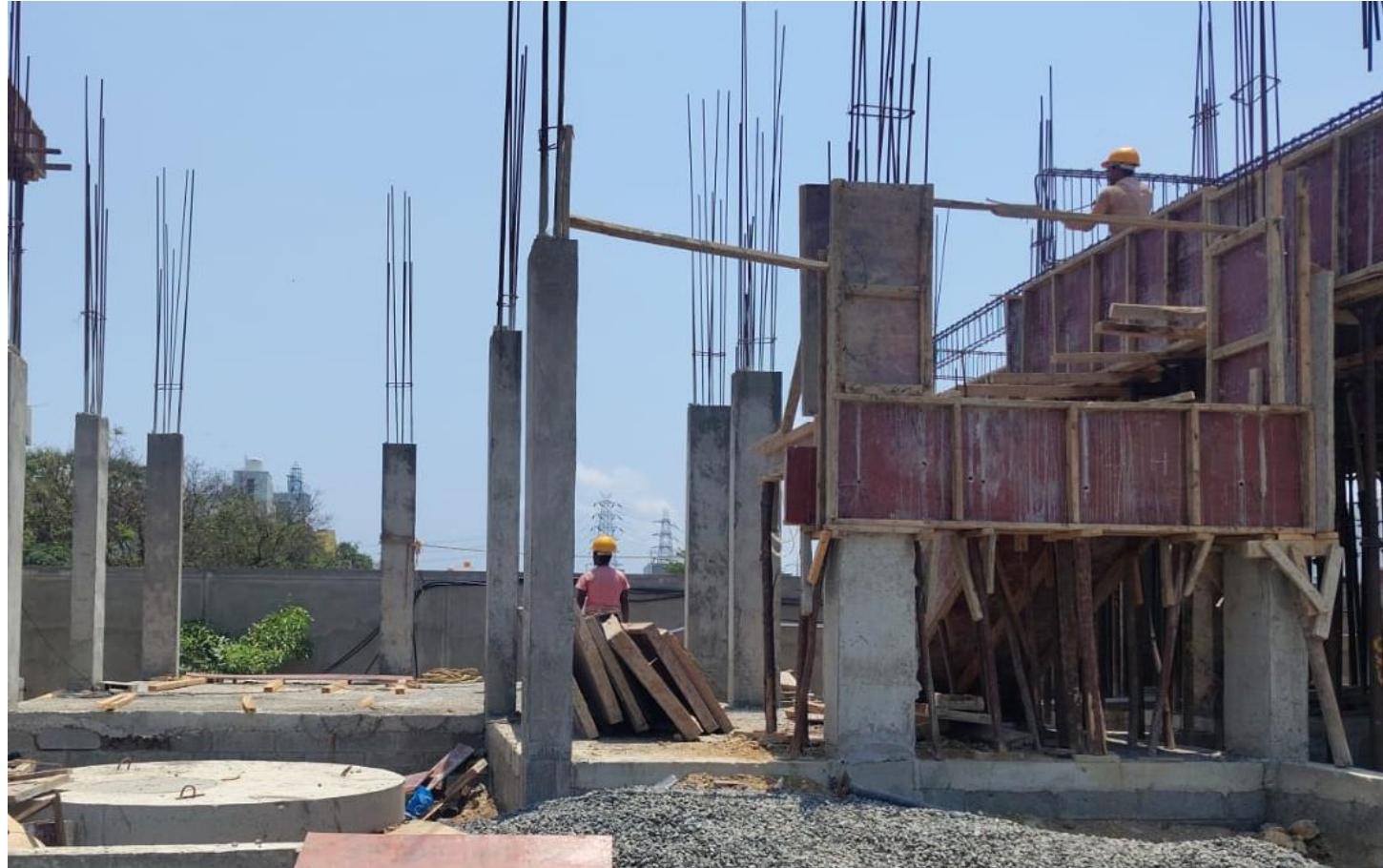
Villa No 23 –GF Roof Slab Shuttering Work In Progress
