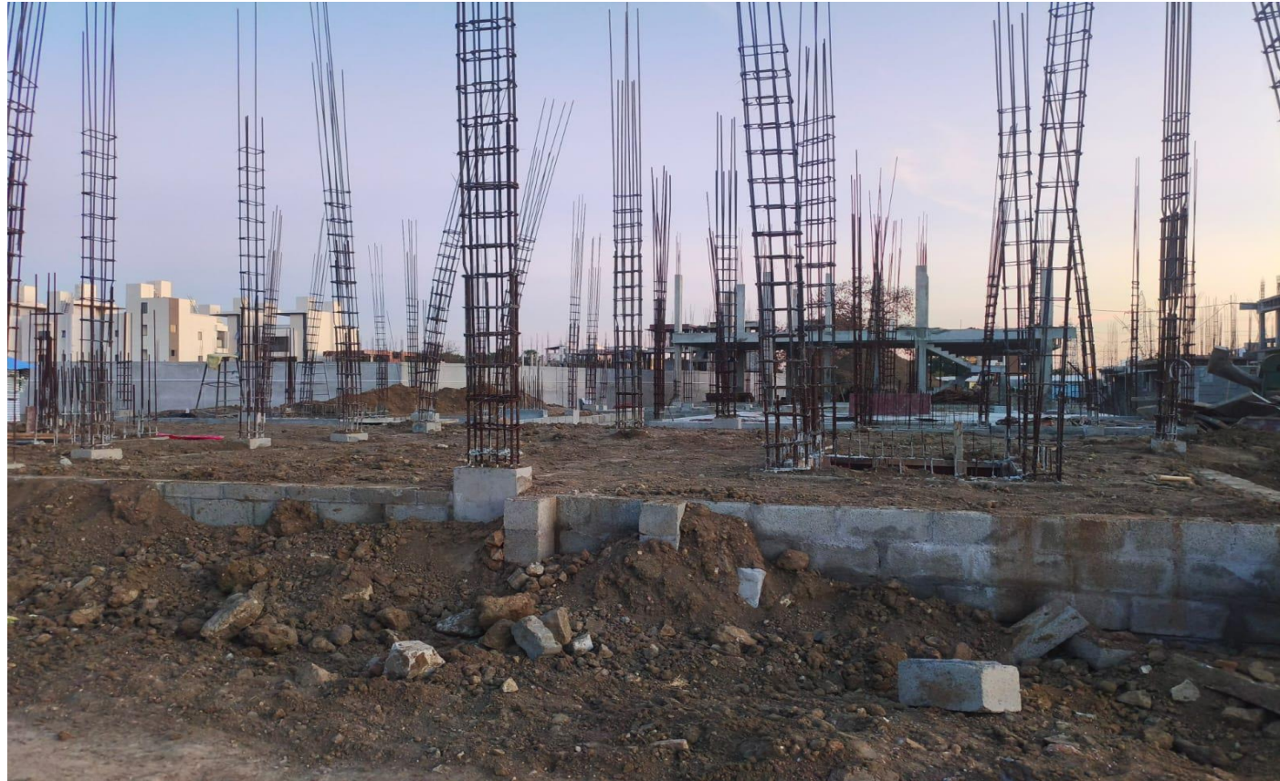
Villa No 104–Basement Back Filling Work Completed
