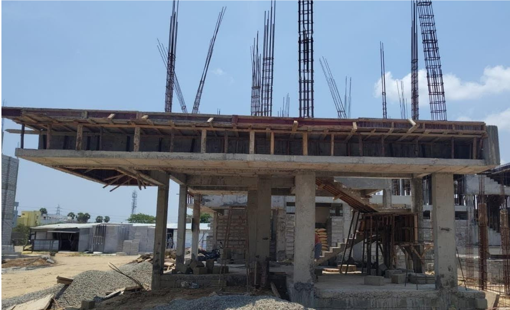
Villa No 33 –FF Column Reinforcement work Completed
