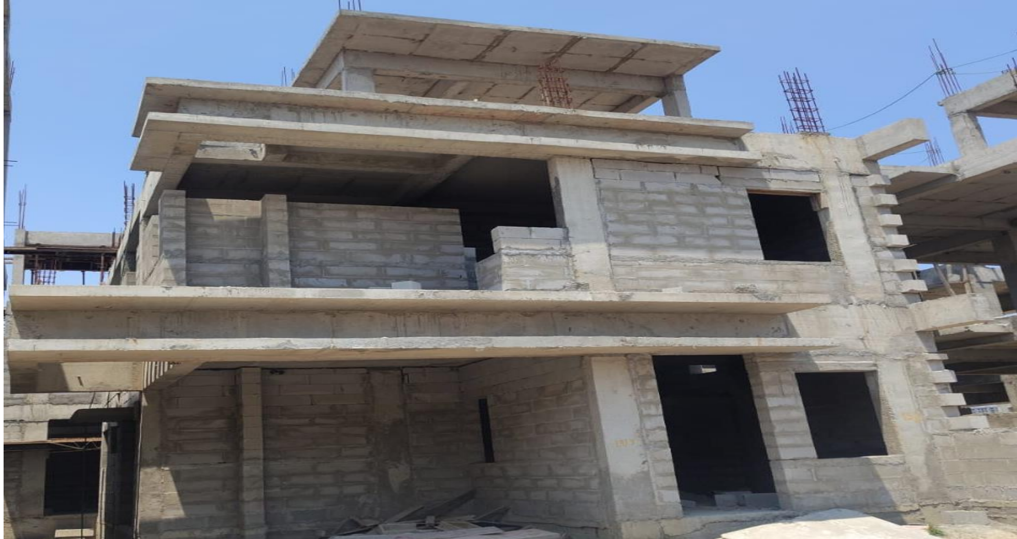
Villa No 52 –FF Block Work In Progress
