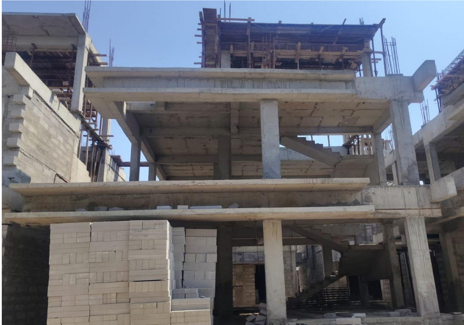
Villa No 57- Head Room Roof Slab Concrete Pouring Completed
