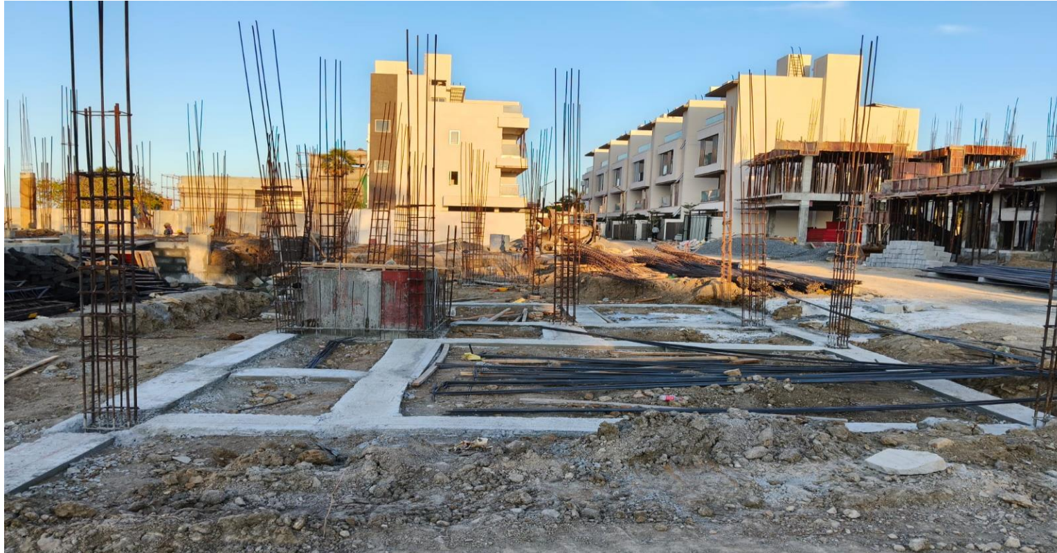
Villa No 116–Plinth Beam PCC Concrete Pouring Completed
