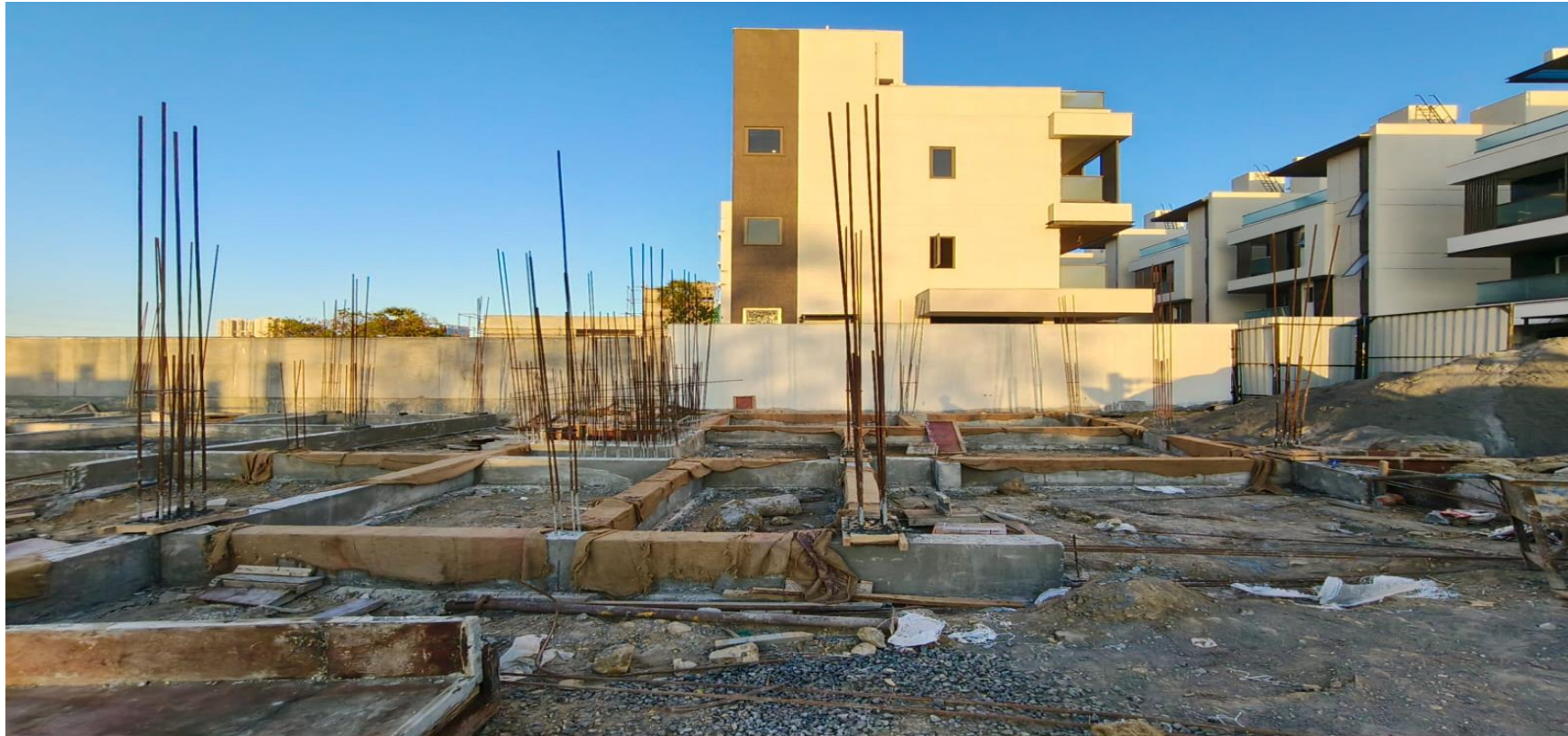
Villa No 123–Plinth Beam Concrete Pouring Completed
