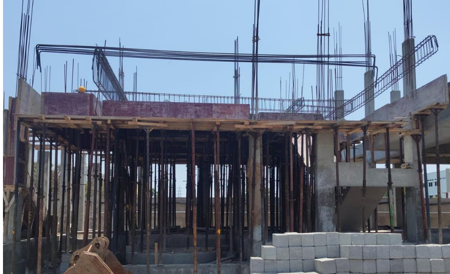
Villa No 24- GF Roof Slab Reinforcement work In Progress
