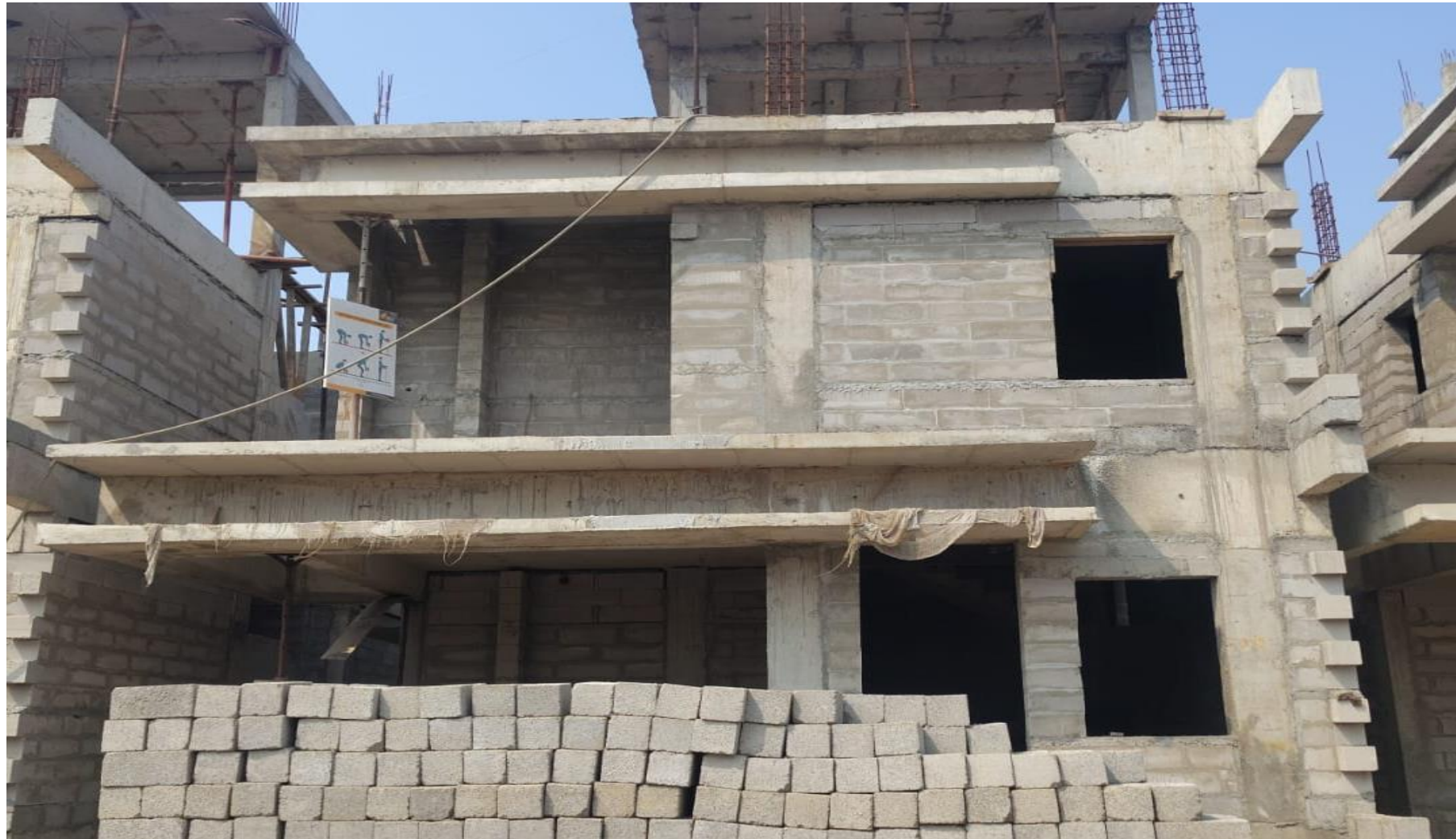
Villa No 49- Parapet Wall Column Reinforcement Work In Progress
