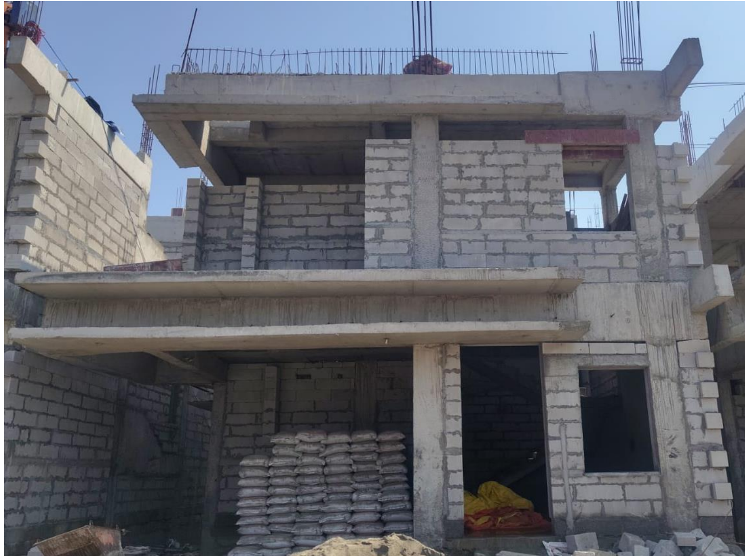
Villa No 76 –FF Block Work In Progress
