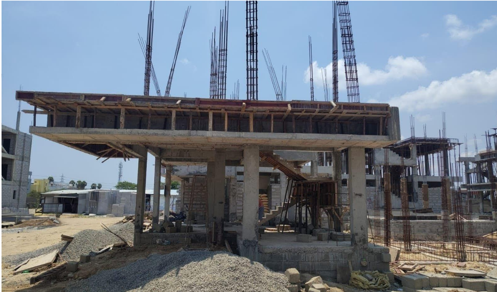
Villa No 33- FF Column Reinforcement work Completed
