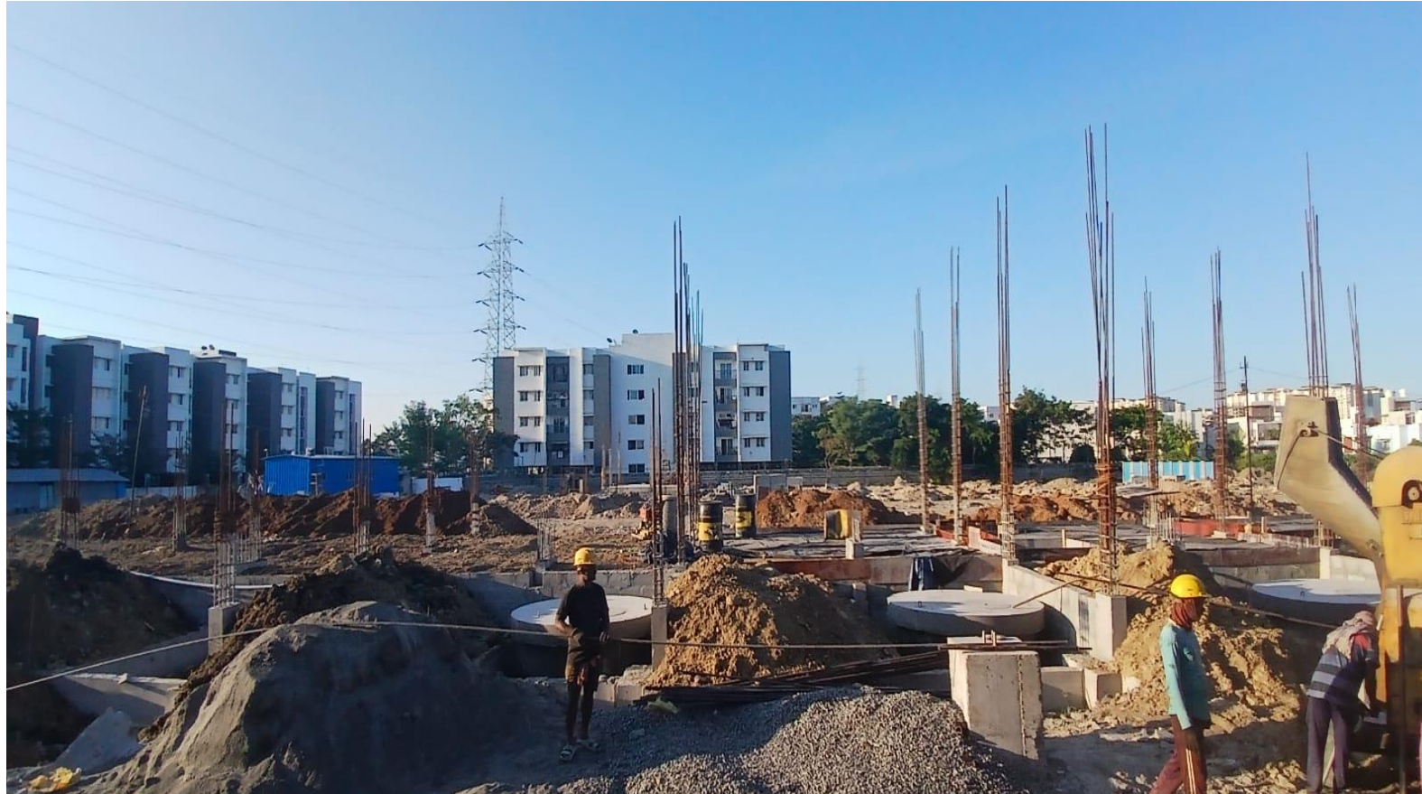
Villa No 88 & 89–GF Column Reinforcement Work In Progress
