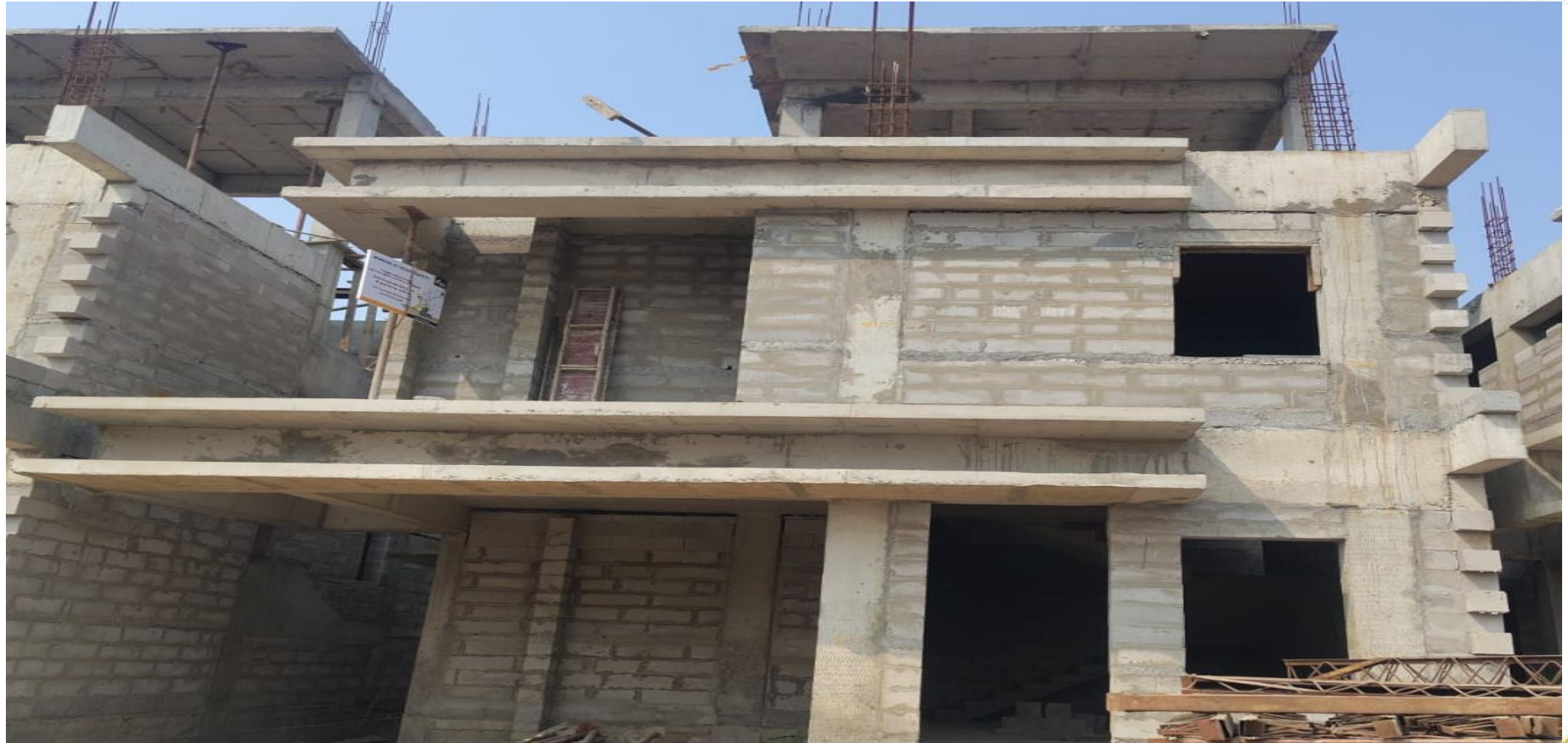
Villa No 50- Head Room Slab Concrete Pouring Completed
