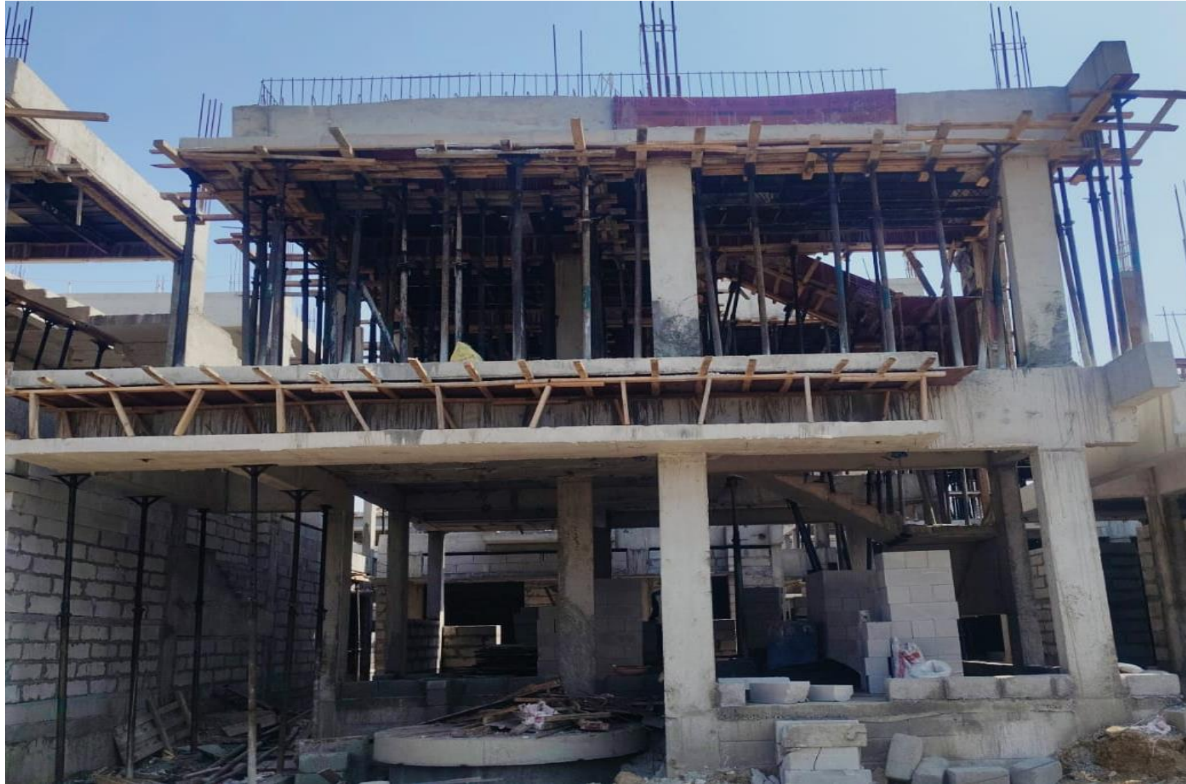
Villa No 78–FF Roof Slab concrete Pouring completed
