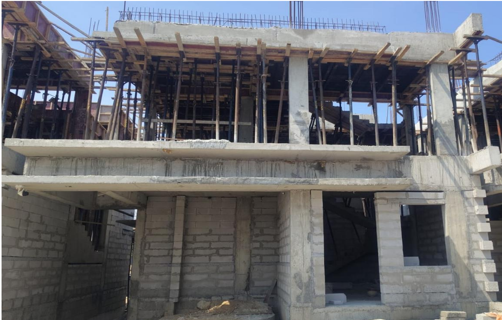
Villa No-64 FF Roof Slab Concrete Pouring Completed
