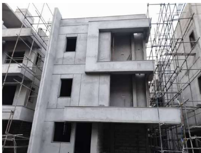
V40 - External Plastering
