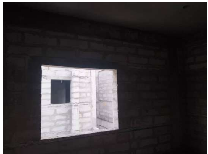
V59 - Completion of Blockwork
