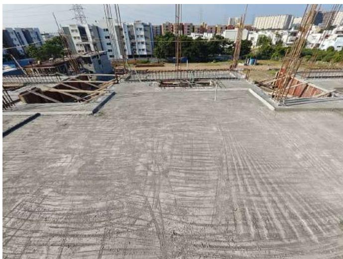
V92- Completion of Staircase Headroom & Part Roof Slab
