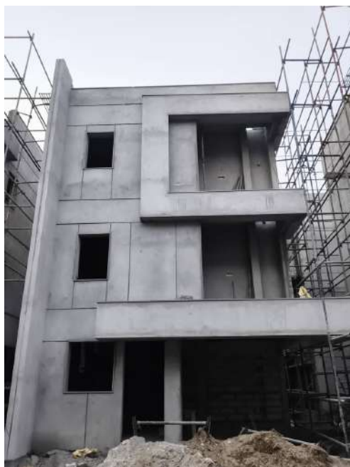
V40 - External Plastering
