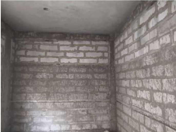
V59 - Completion of Blockwork
