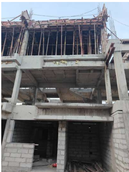
V96 - Staircase Headroom with Part Roof Slab & Beam Concreting
