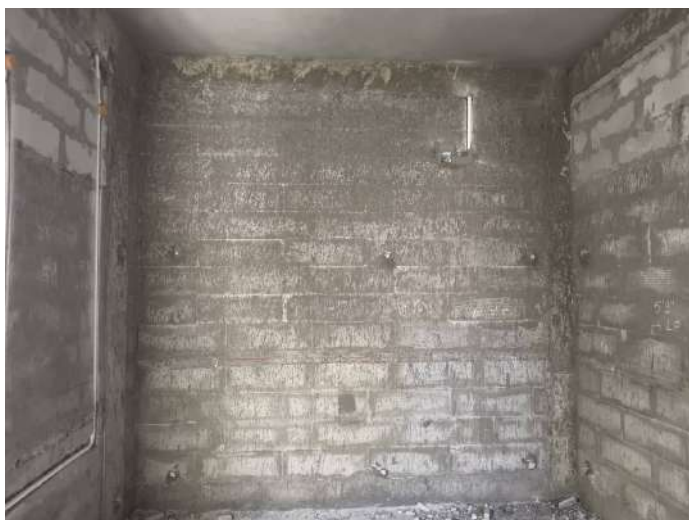
V57 - Completion of Blockwork
