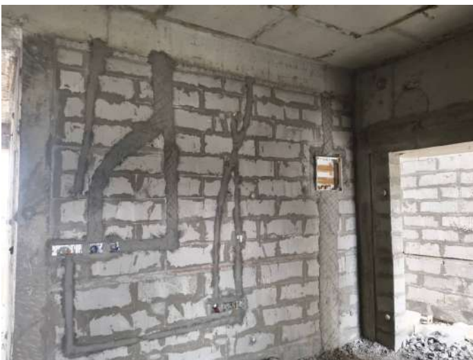
V23 - Completion of Blockwork
