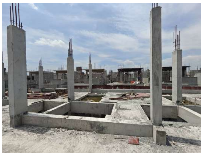
V91 - Stair Head Room Column Concreting
