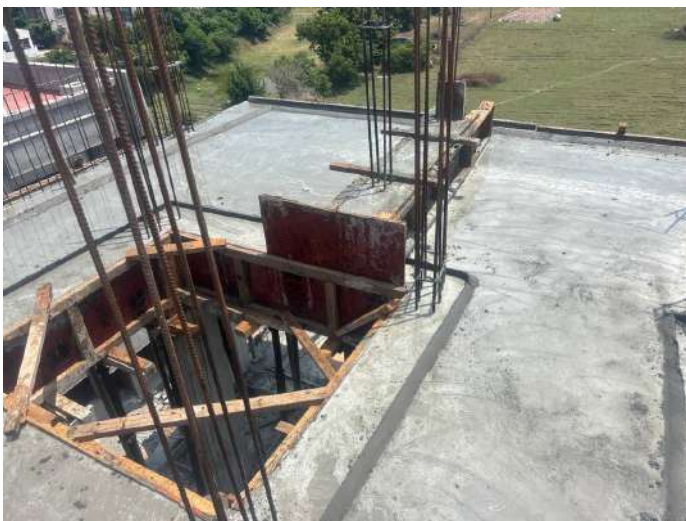
V104 - Stair Head Room Roof Slab & Beam Concreting
