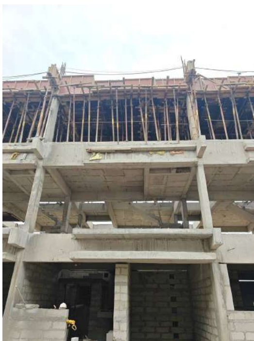
V95 - Completion of Staircase Headroom with Part roof slab
