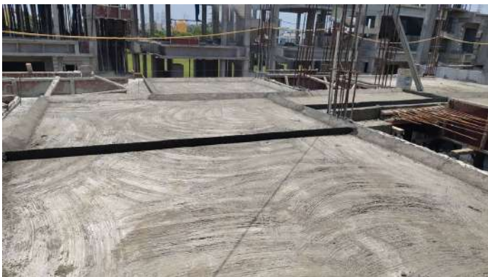
V117 - Completion of First Floor Roof Slab
