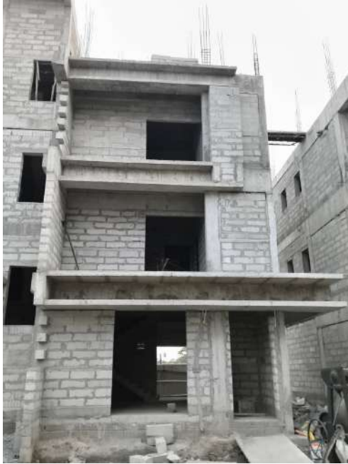
V28 - Installation of Wall chasing & Electrical conduits
