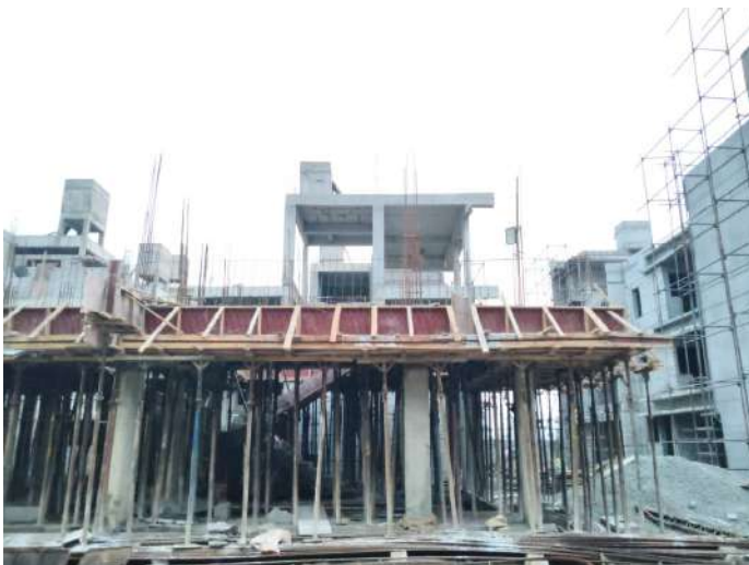
V35 - Ground Floor Roof Slab & Beam Concreting
