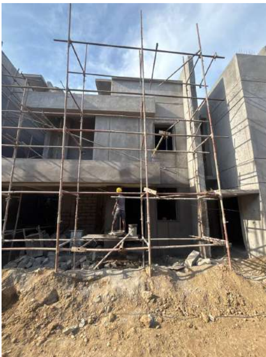
V70 - External Plastering
