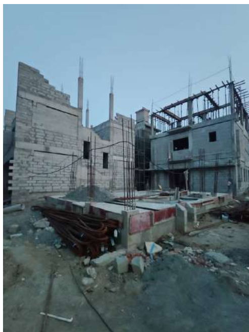
V82 - Ground Floor Column Concreting
