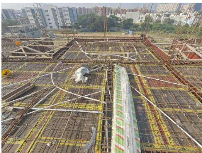
V95 - Staircase Headroom with Part Roof Slab - Shuttering, Reinforcement
