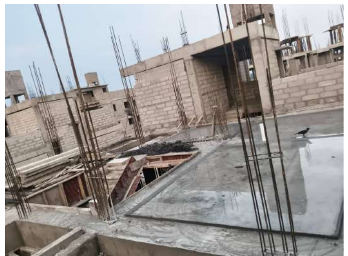
V34 - First Floor Roof Slab & Beam Concreting
