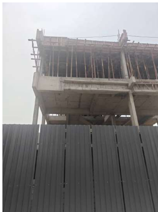
V97 - Completion of Staircase Headroom with Part roof slab
