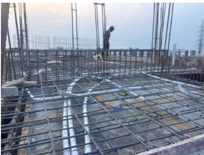
V107 - Stair Head Room Roof Slab & Beam - Shuttering, Reinforcement
