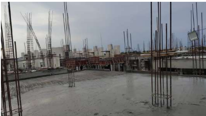
V113 - Completion of Second Floor Roof Slab
