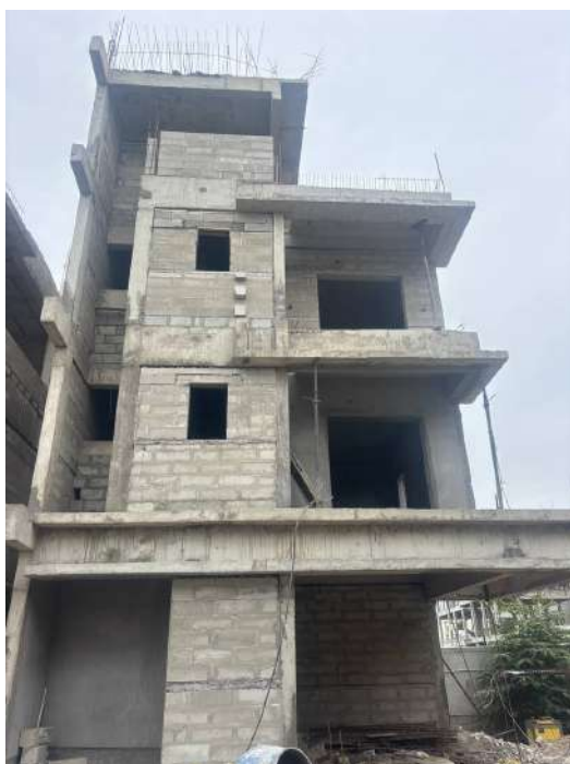
V108 - Completion of Blockwork
