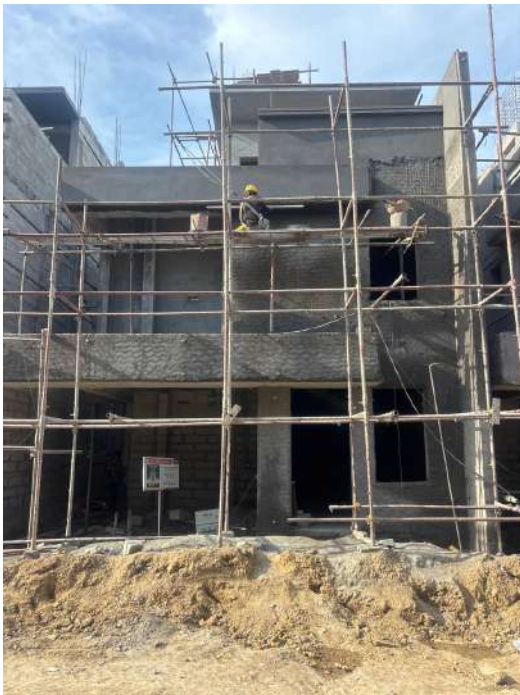
V69 - External Plastering
