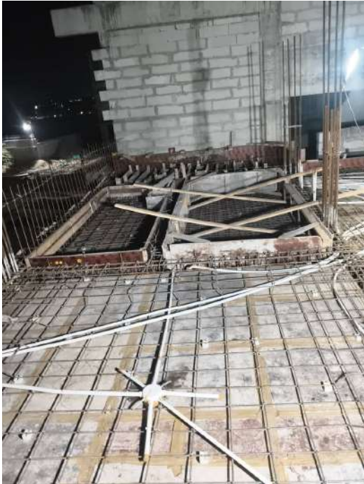
V34 - Ground Floor Roof Slab & Beam - Shuttering, Reinforcement
