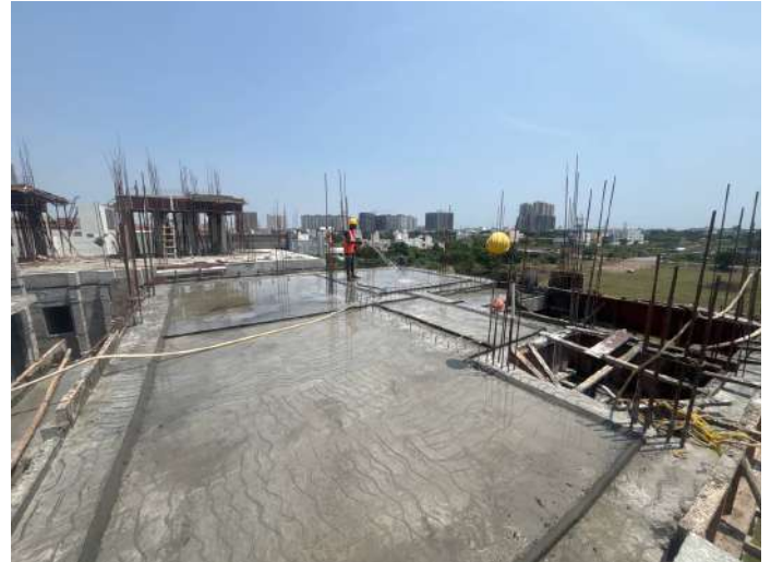
V103 - SF- Roof Slab & Beam Concreting
