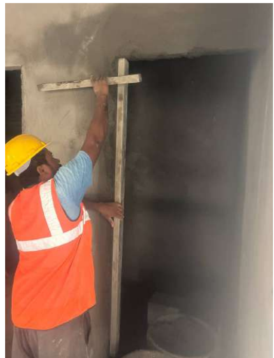
V106 - Internal Plastering
