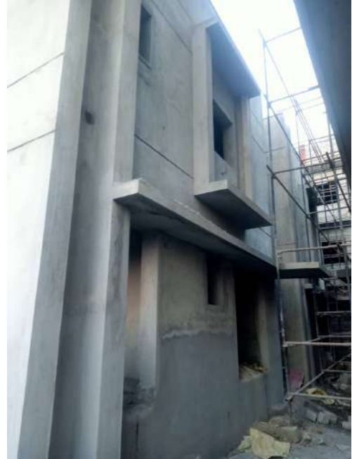
V45 - External Plastering
