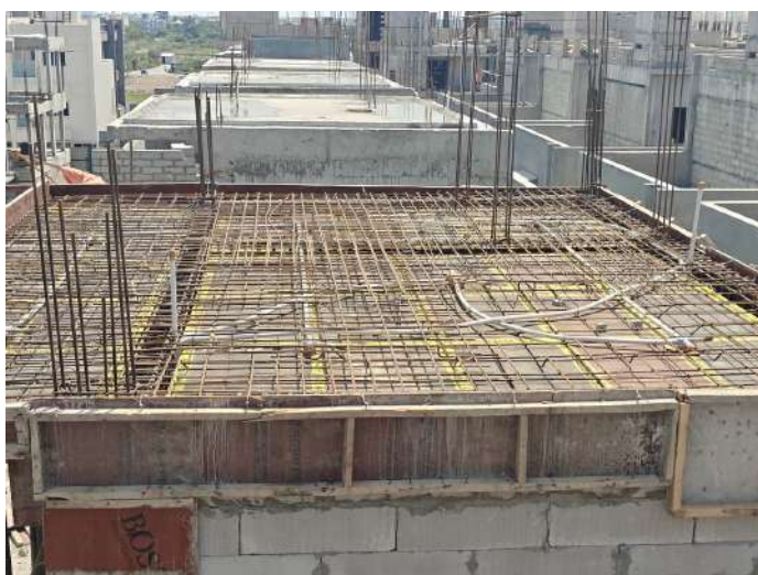
V79 - Stair Head Room Roof Slab & Beam - Electrical works
