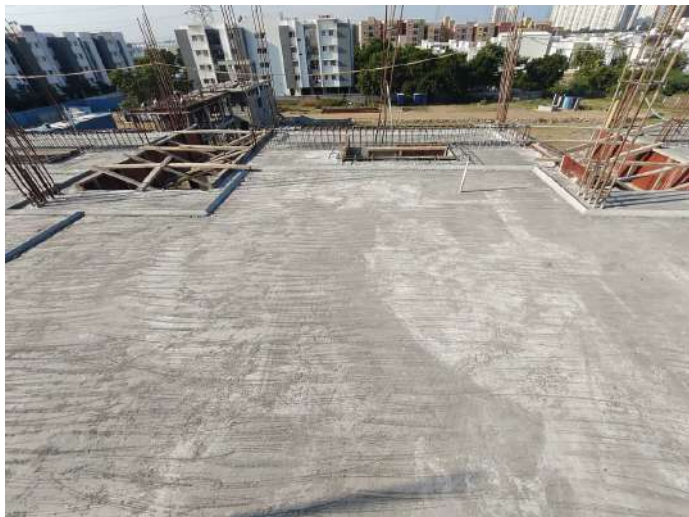
V91 - Stair Head Room Roof Slab & Beam Concreting
