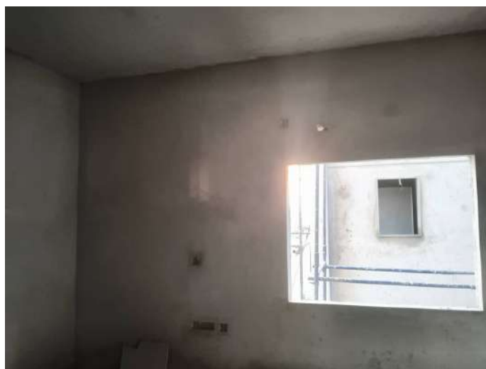
V30 - Internal Plastering
