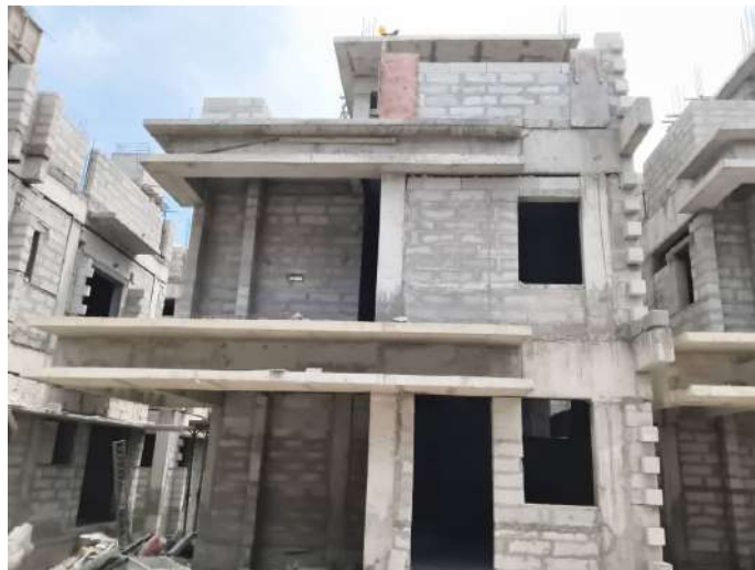
V56 - Completion of Blockwork
