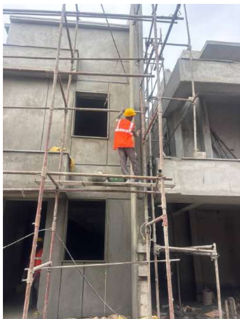
V68 - External Plastering
