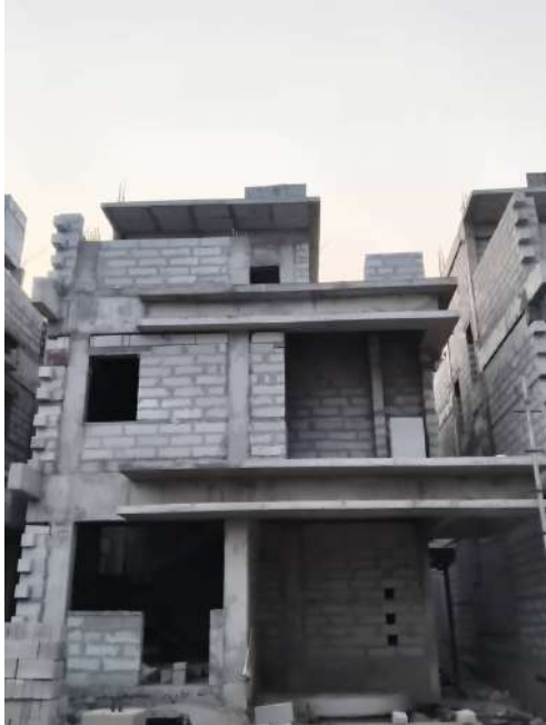
V54 - Instllation of Wall chasing & Electrical conduits
