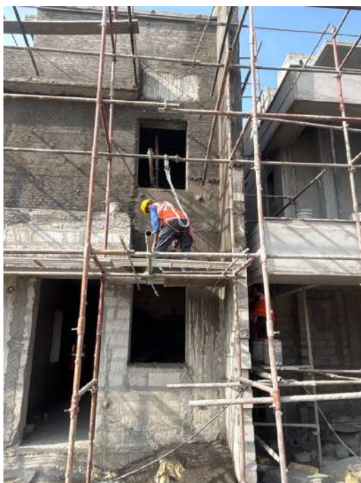
V64 - External Plastering
