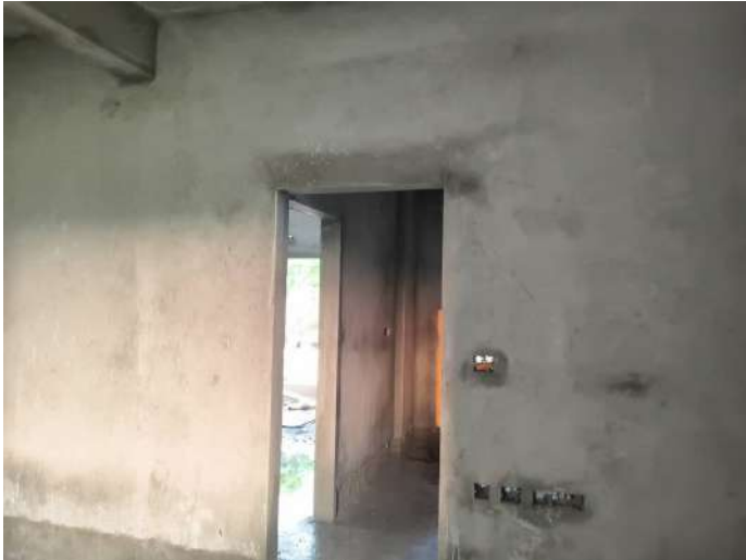
V30 - Internal Plastering
