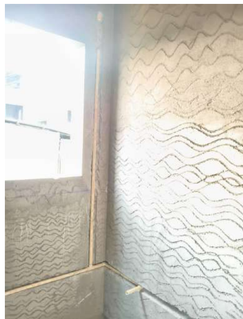
V29 - Internal Plumbing Core Cutting & Wall chasing
