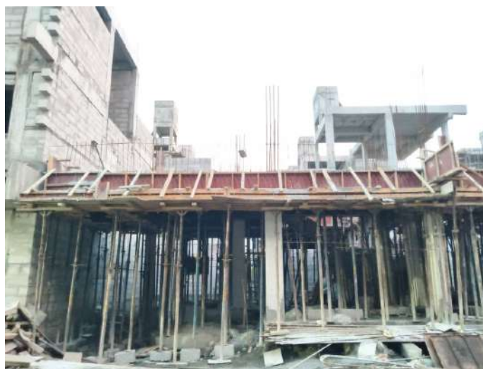
V34 - Completion of Ground Floor Roof Slab
