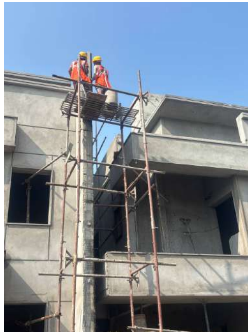
V64 - External Plastering
