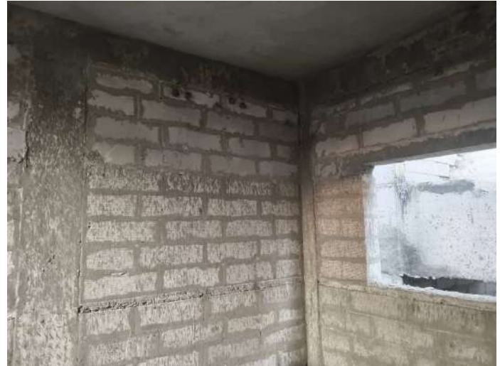
V59 - Completion of Blockwork
