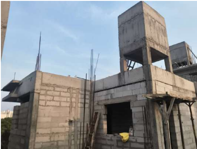
V31 - Completion of Staircase Headroom with Part roof slab
