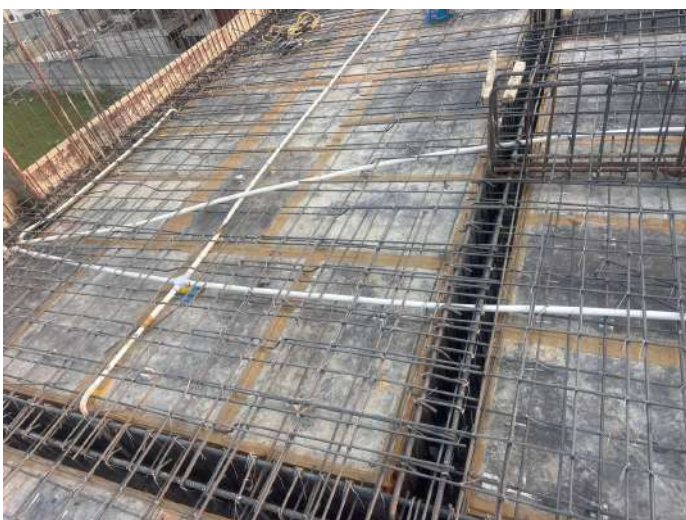
V103 - Stair Head Room Roof Slab & Beam - Electrical works
