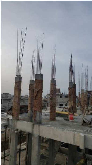
V110 - Stair Head Room Column Concreting
