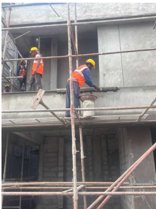
V65 - External Plastering
