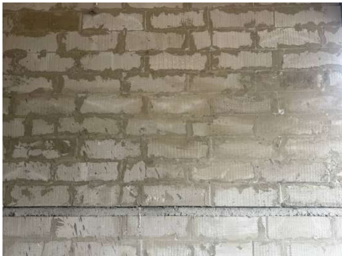
V108 - Completion of Blockwork
