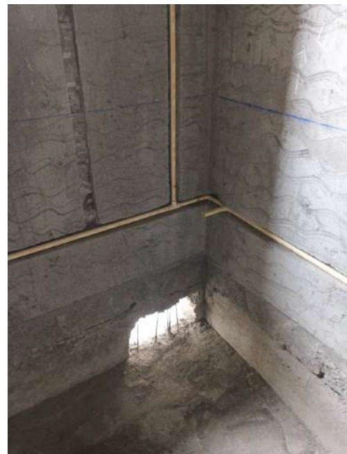
V39 - Internal Plumbing Core Cutting & Wall chasing
