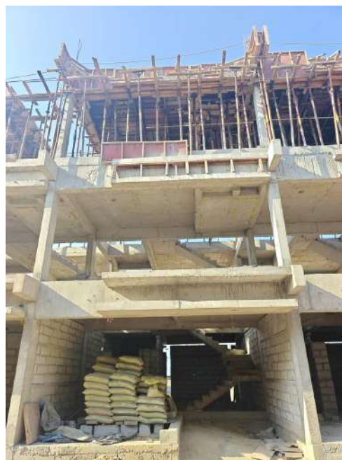
V89 - Stair Head Room Roof Slab & Beam Concreting
