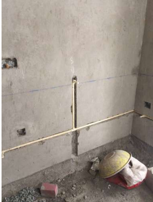
V37 - Internal Plumbing Core Cutting & Wall chasing
