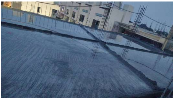
V117 - Completion of Second Floor Roof Slab
