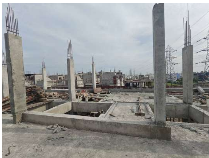
V84 - Stair Head Room Column Concreting
