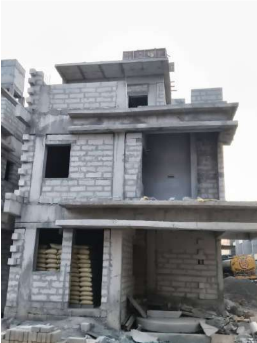
V55 - Instllation of Wall chasing & Electrical conduits
