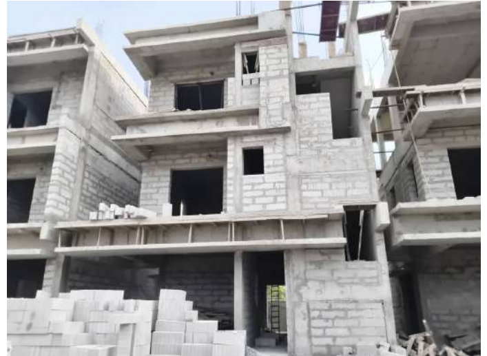
V23 - Completion of Blockwork
