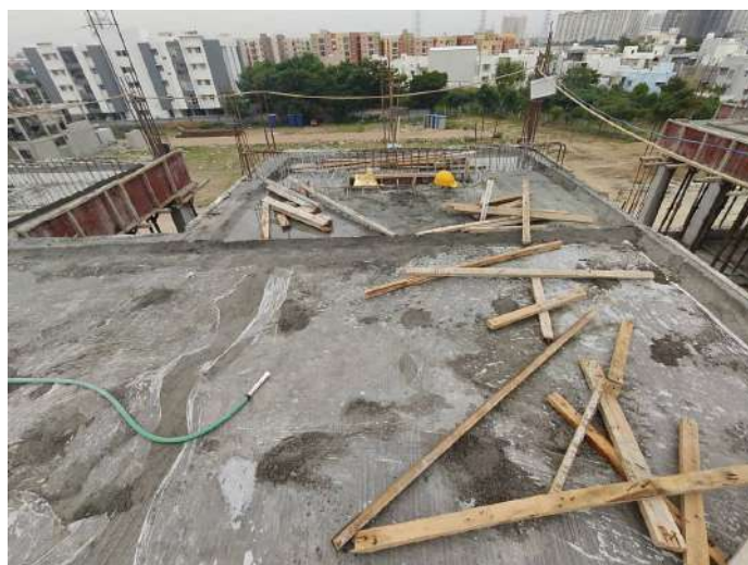
V96 - Completion of Staircase Headroom with Part roof slab
