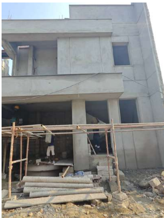
V81 - External Plastering
