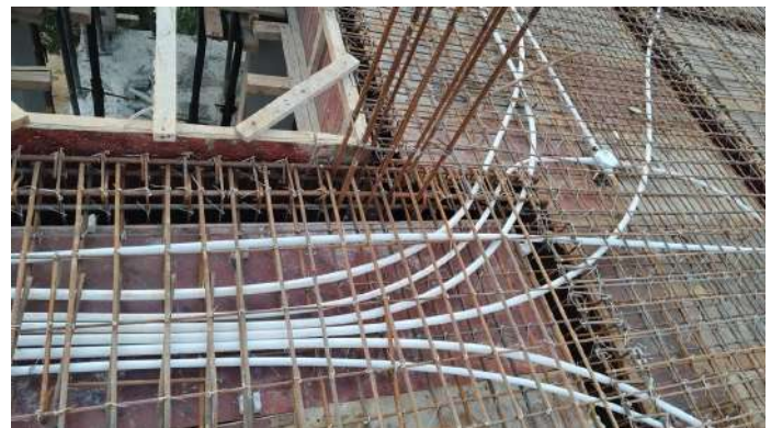
V109 - SF- Roof Slab & Beam - Electrical works
