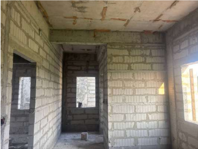
V23 - Completion of Blockwork
