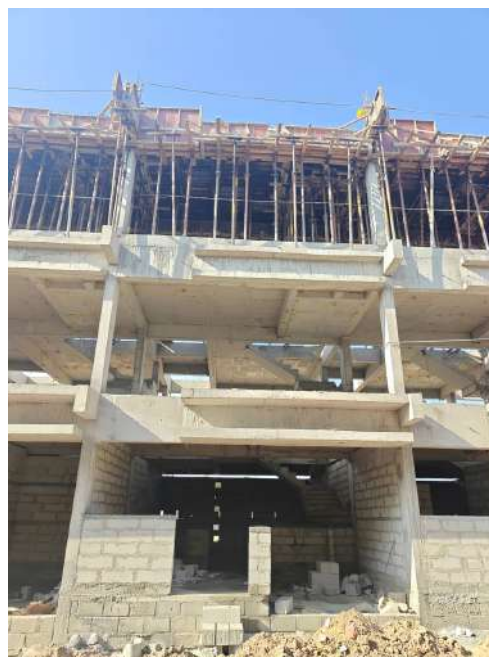
V92- Completion of Staircase Headroom & Part Roof Slab
