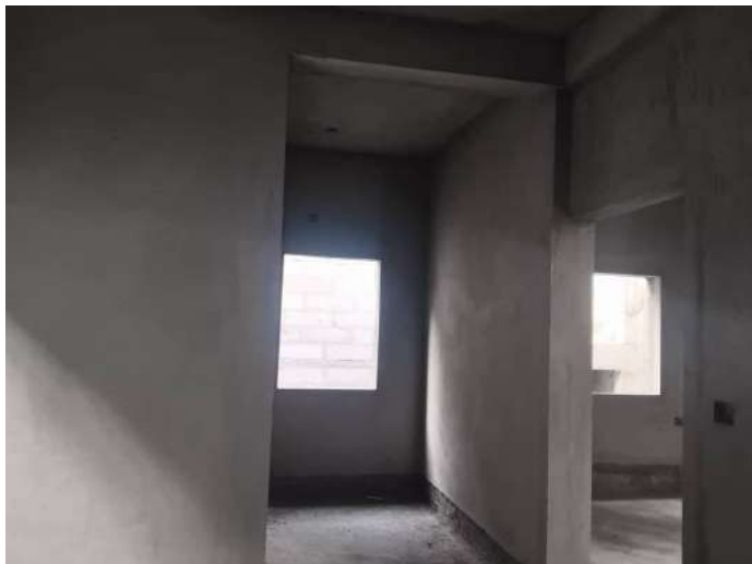
V31 - Internal Plastering
