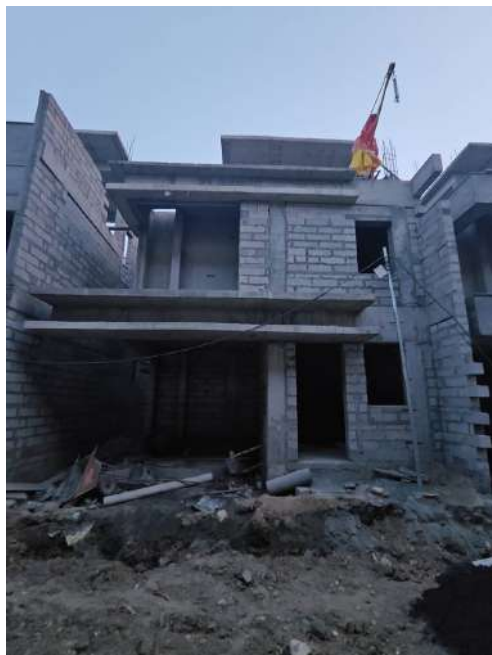
V77 - External Plastering
