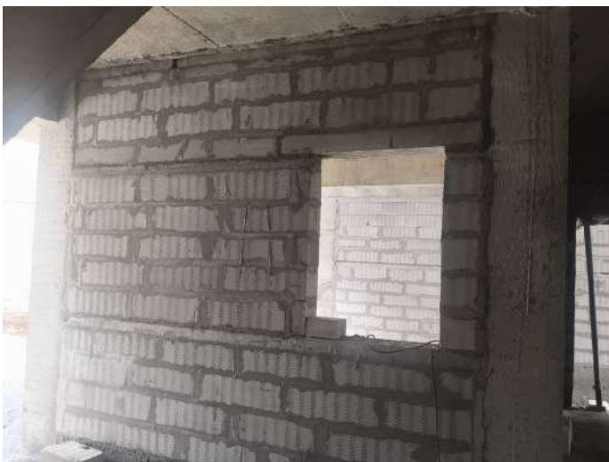
V27 - Completion of Blockwork
