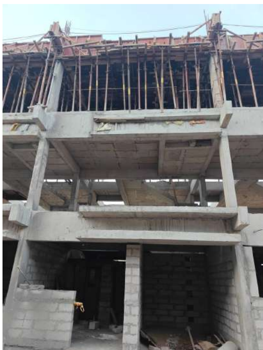
V95 - Staircase Headroom with Part Roof Slab Concreting
