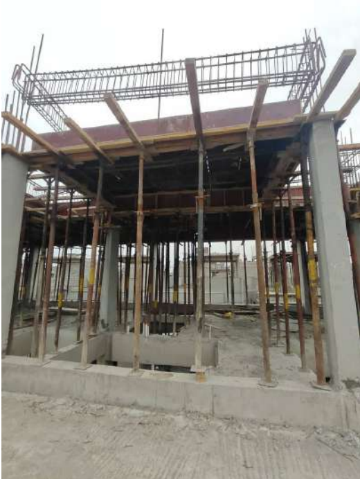
V92 - Stair Head Room Roof Slab & Beam - Shuttering, Reinforcement
