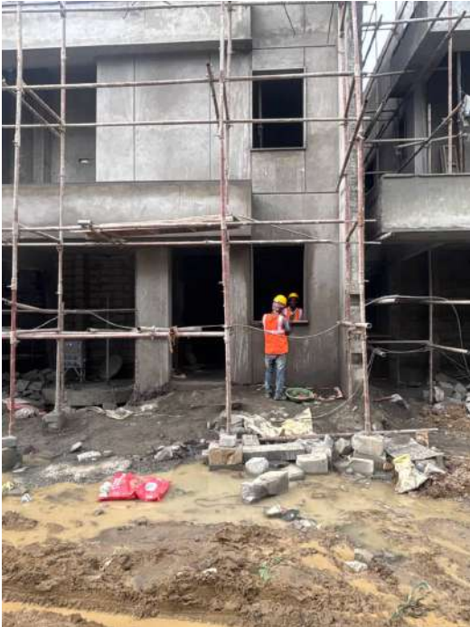
V66 - External Plastering
