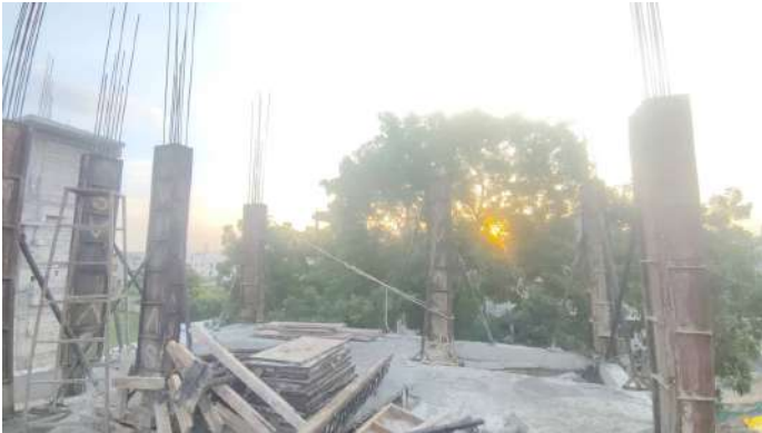
V109 - SF- Column Concreting
