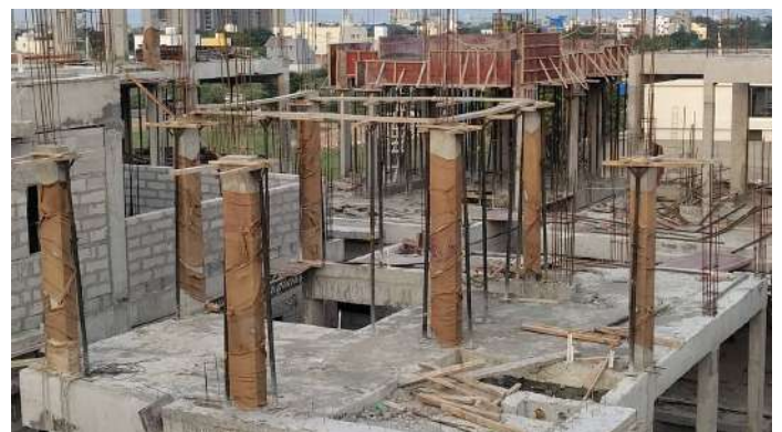
V115 - Staircase Head Room Column Concreting
