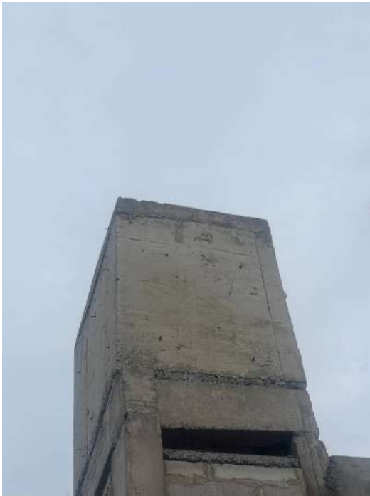
V66 - OHT Cover Slab Concreting
