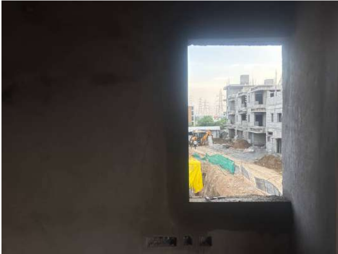
V108 - Internal Plastering
