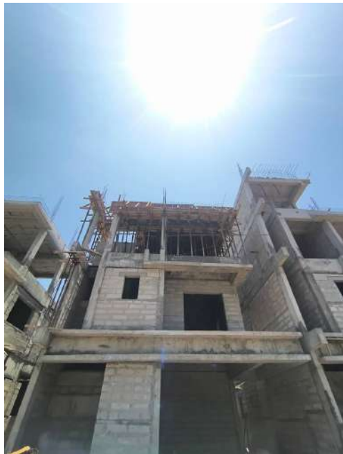
V107 - Completion of Second Floor Roof Slab
