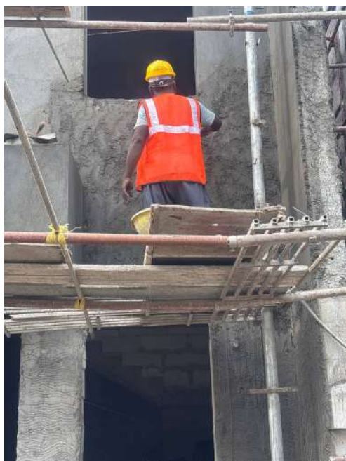
V67 - External Plastering
