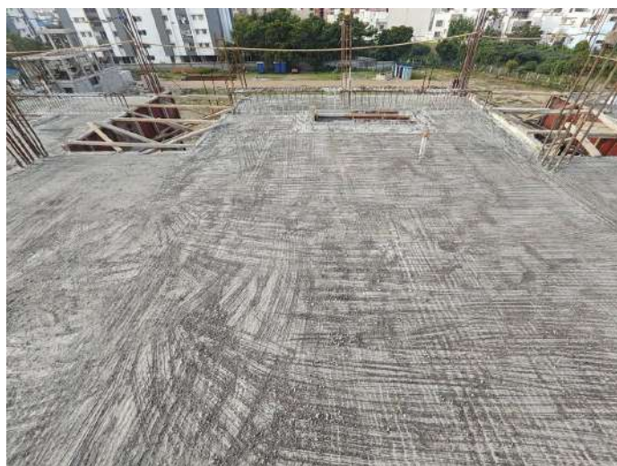
V95 - Staircase Headroom with Part Roof Slab Concreting
