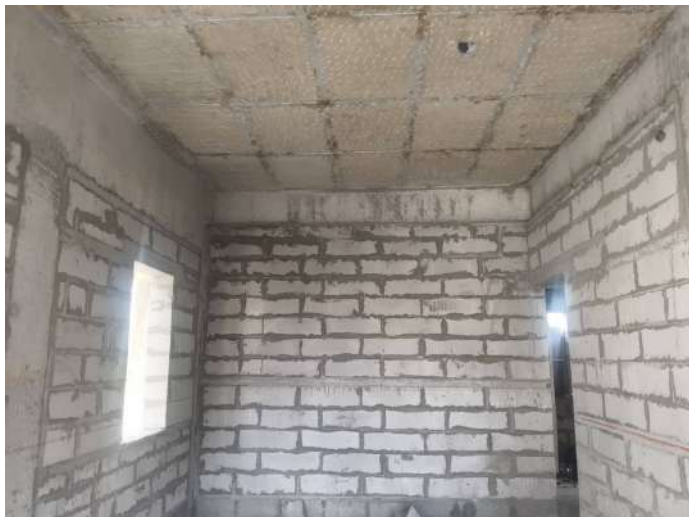
V27 - Completion of Blockwork
