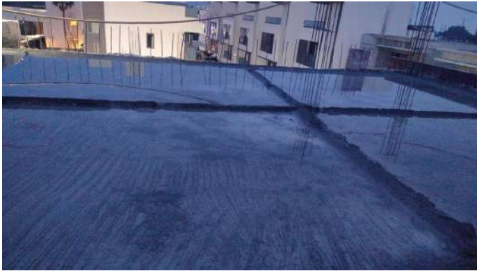
V117 - SF- Roof Slab & Beam Concreting
