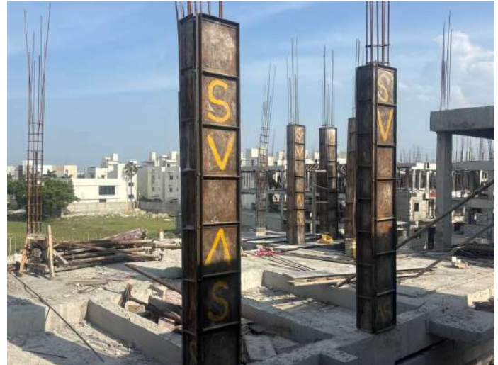
V103 - SF- Column Concreting
