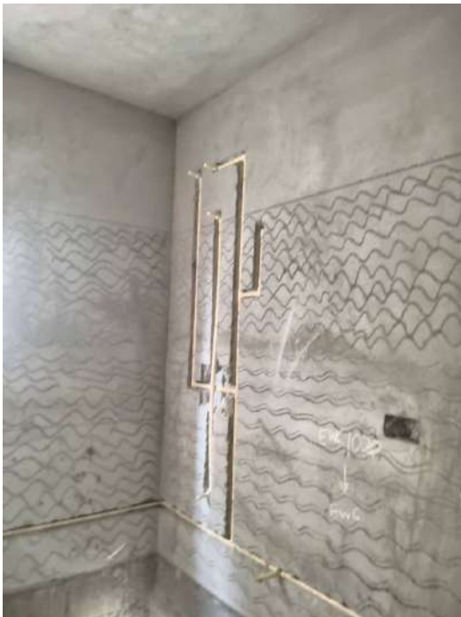
V29 - Instllation of Internal Plumbing
