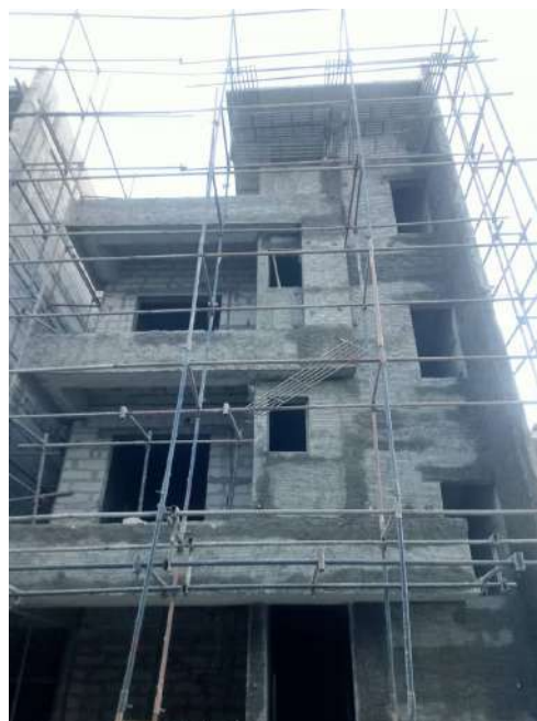
V43 - External Plastering
