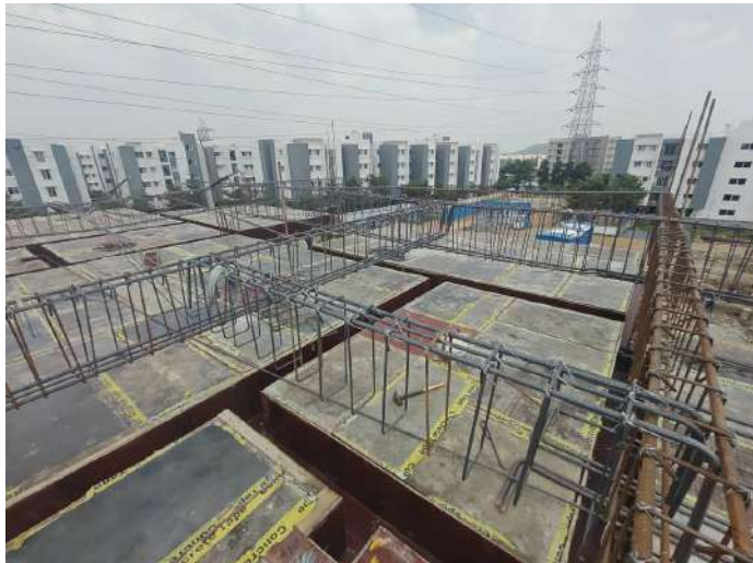
V84 - Stair Head Room Roof Slab & Beam - Shuttering, Reinforcement
