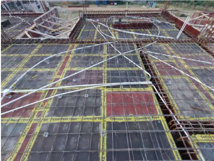
V93 - Stair Head Room Roof Slab & Beam - Electrical works
