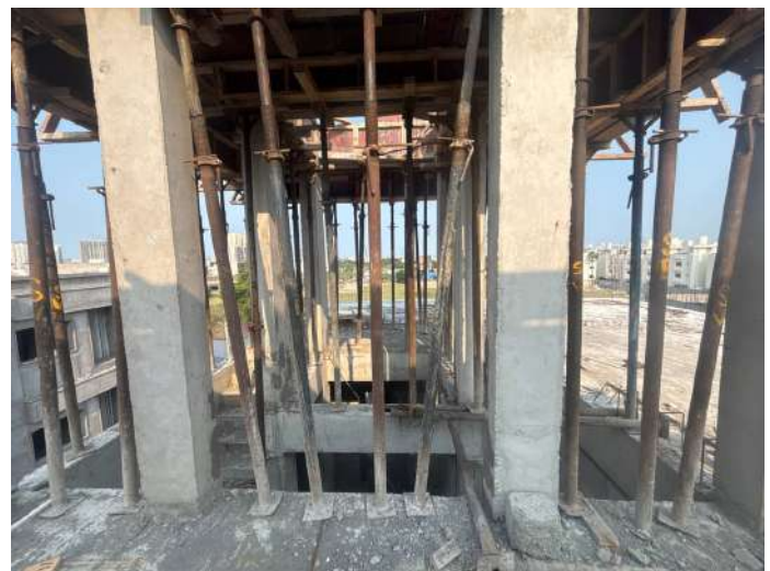
V104 - Stair Head Room Column Concreting
