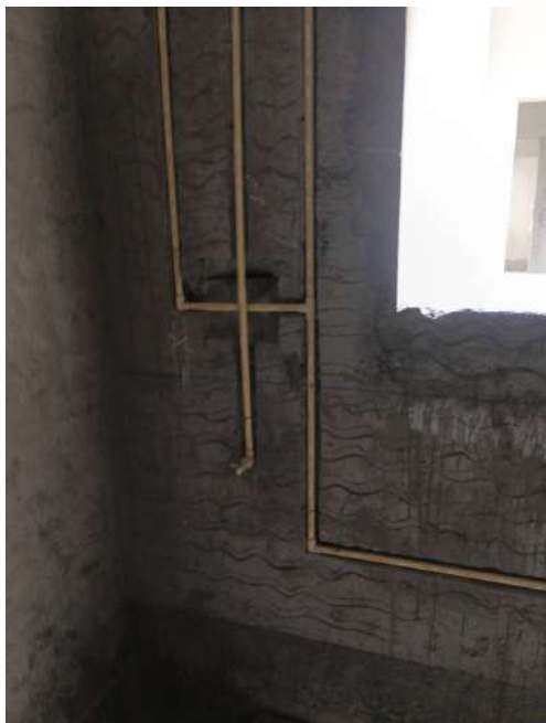
V39 - Internal Plumbing Core Cutting & Wall chasing
