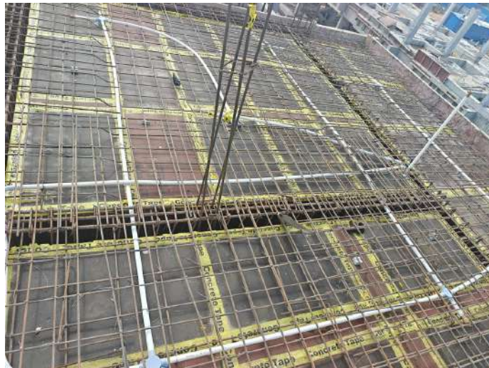
V78 - Stair Head Room Roof Slab & Beam - Electrical works
