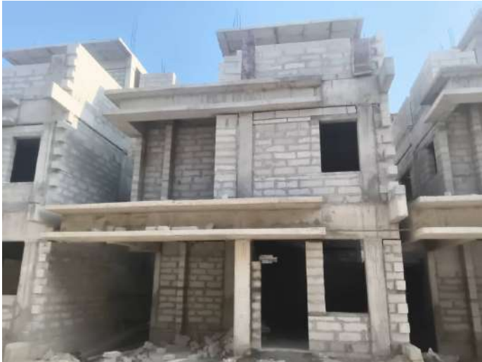
V57 - Completion of Blockwork
