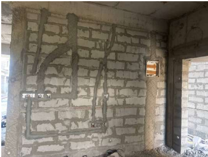
V23 - Completion of Blockwork
