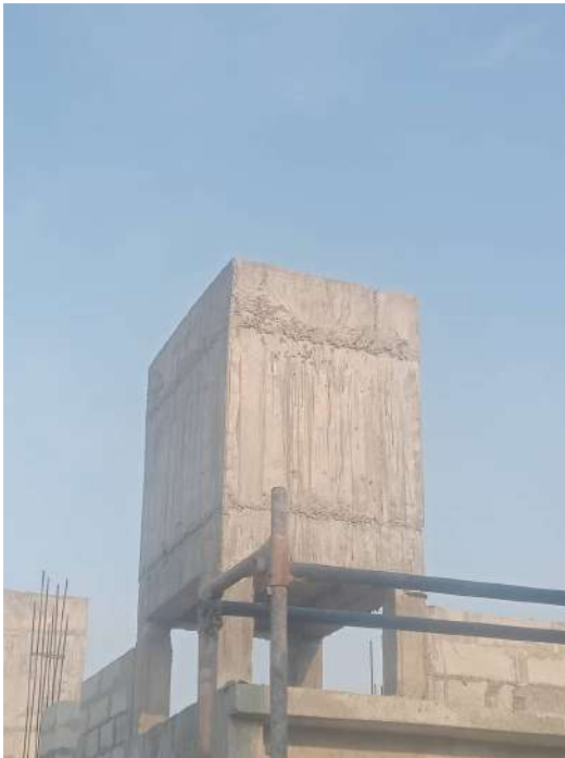
V47 - OHT Cover Slab Concreting
