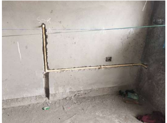
V29 - Instllation of Internal Plumbing
