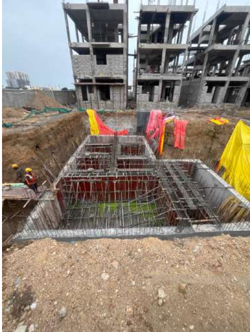
STP - Civil works
