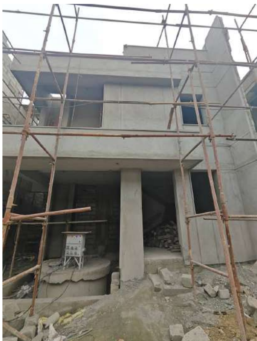
V80 - External Plastering
