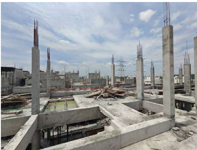
V87 - Stair Head Room Column Concreting
