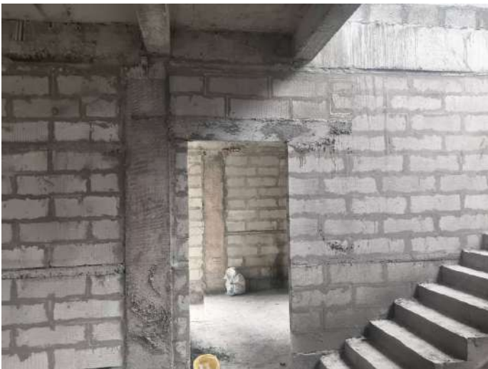
V36 - Completion of Blockwork
