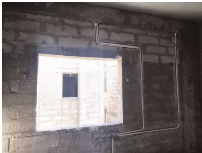
V56 - Instllation of Wall chasing & Electrical conduits
