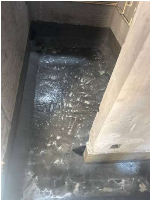
V70 - Toilet Waterproofing
