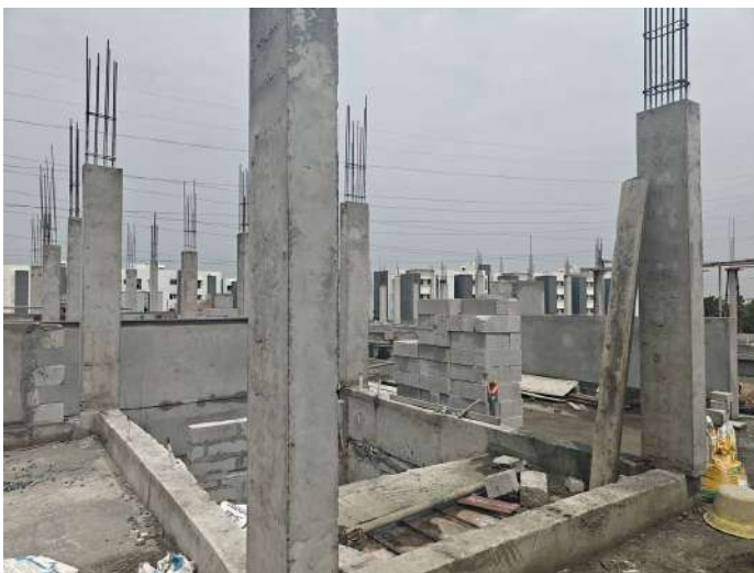
V79 - Stair Head Room Column Concreting
