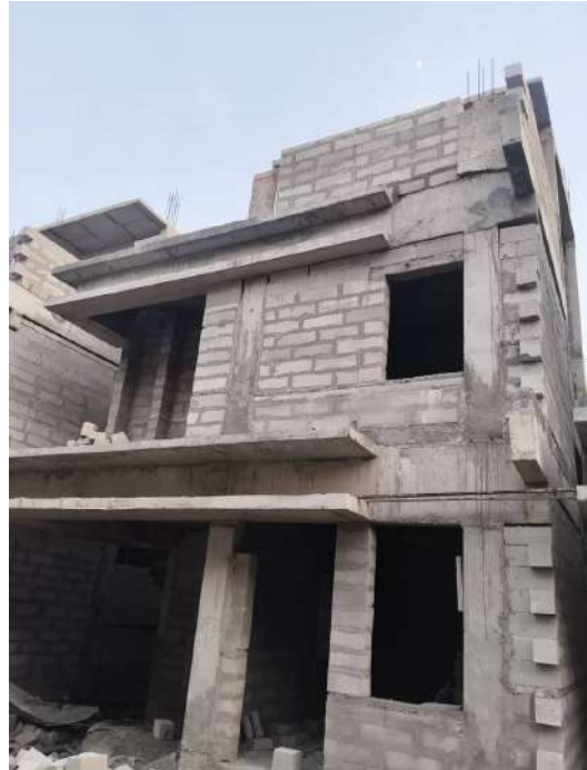
V58 - Completion of Blockwork
