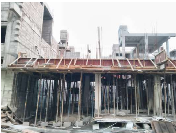
V34 - Ground Floor Roof Slab & Beam Concreting
