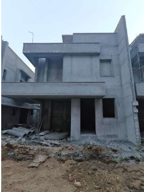
V74 - External Plastering
