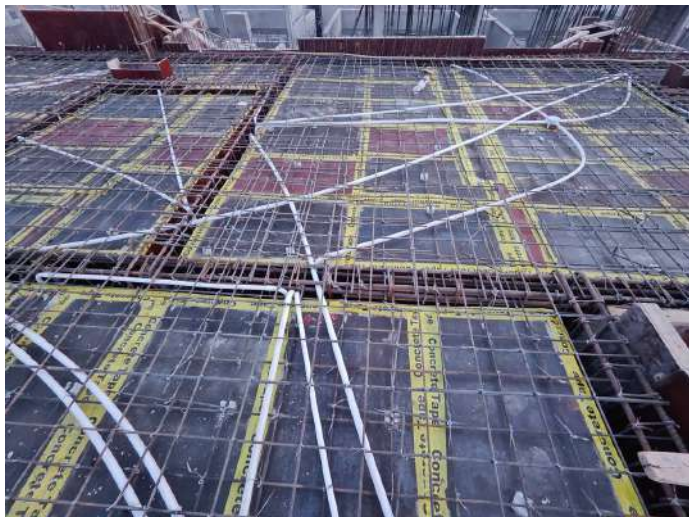
V89 - Stair Head Room Roof Slab & Beam - Electrical works
