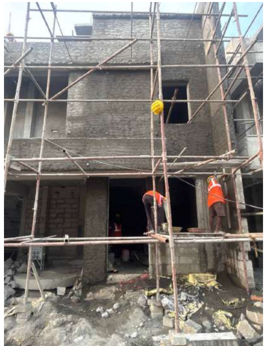
V66 - External Plastering
