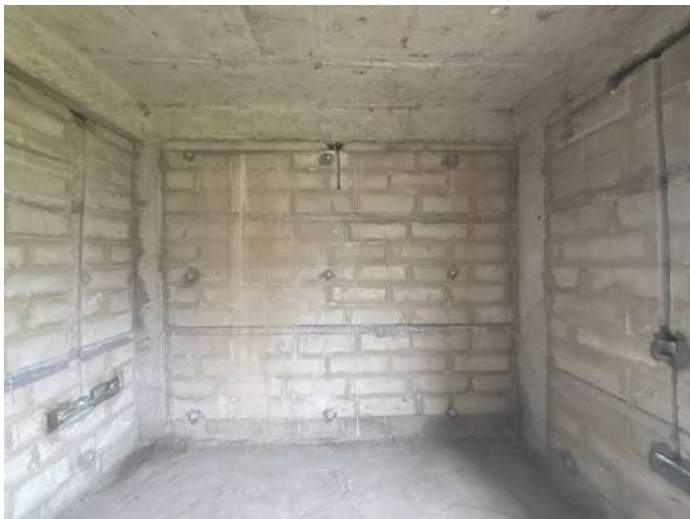
V108 - Completion of Blockwork
