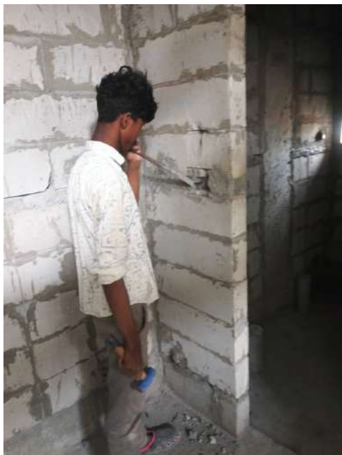
V98 - Installation of Wall chasing & Electrical conduits
