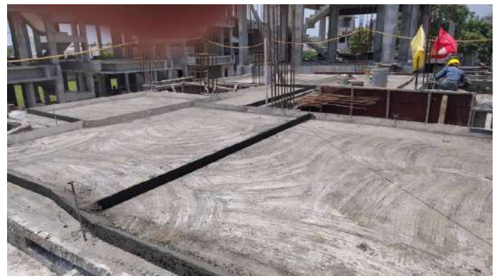
V117 - First Floor Roof Slab & Beam Concreting
