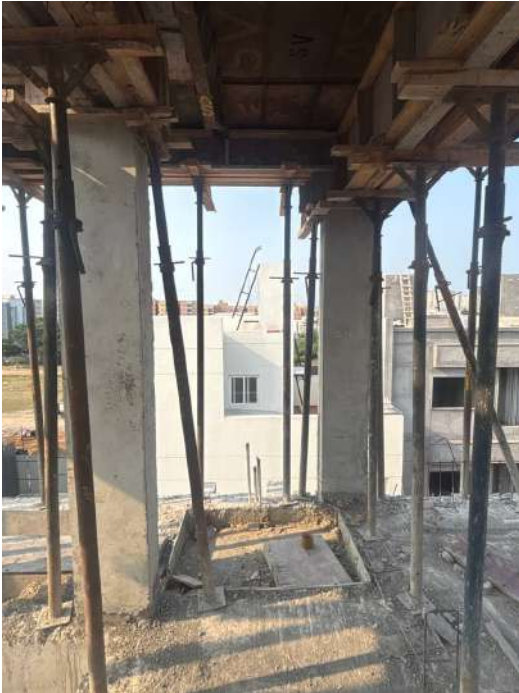
V105 - Stair Head Room Column Concreting
