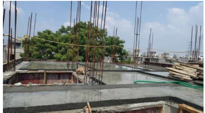
V109 - SF- Roof Slab & Beam Concreting
