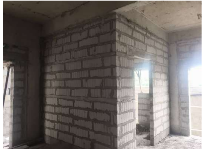
V27 - Completion of Blockwork
