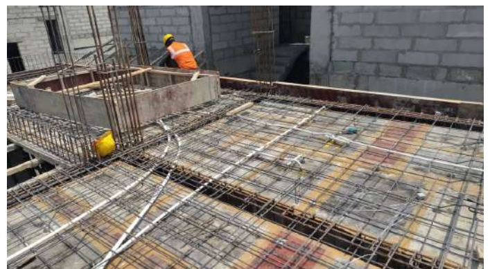
V117 - SF- Roof Slab & Beam - Shuttering, Reinforcement
