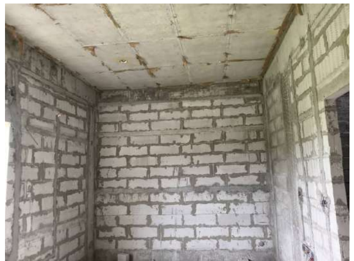
V23 - Completion of Blockwork
