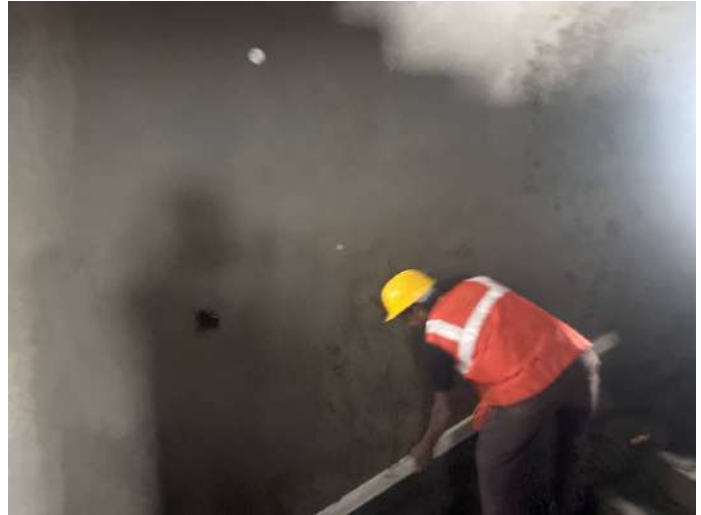
V106 - Internal Plastering
