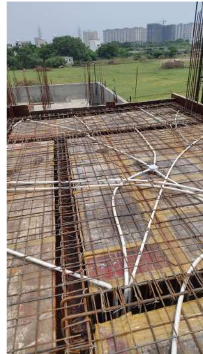
V123 - Ground Floor Roof Slab & Beam - Electrical works
