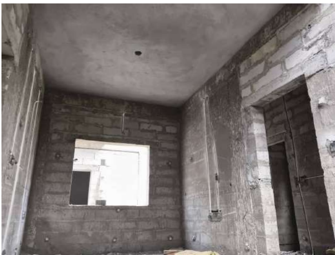
V56 - Completion of Blockwork
