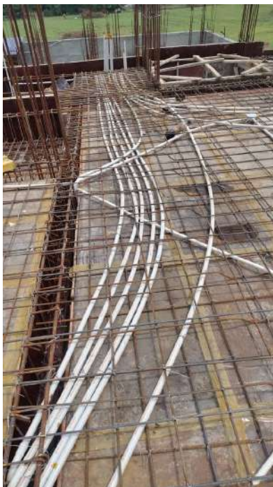
V123 - Ground Floor Roof Slab & Beam - Electrical works
