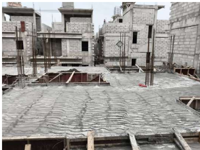
V34 - Ground Floor Roof Slab & Beam Concreting
