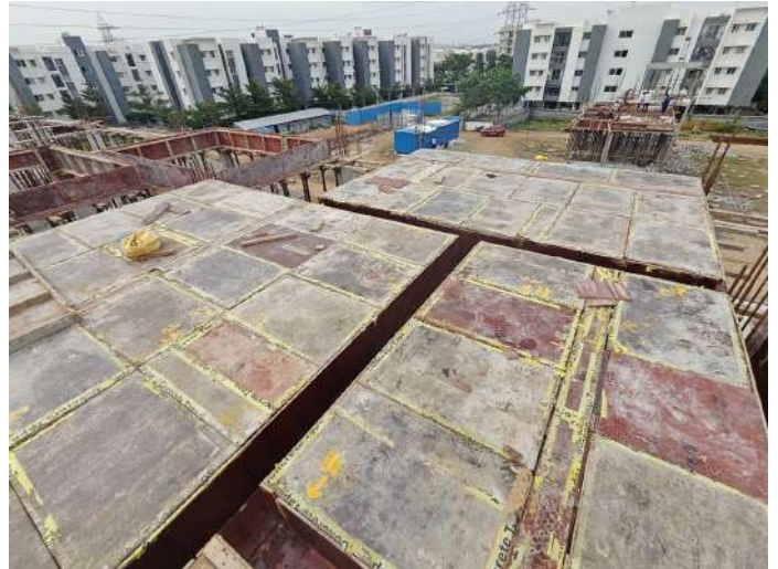
V87 - Stair Head Room Roof Slab & Beam - Shuttering, Reinforcement
