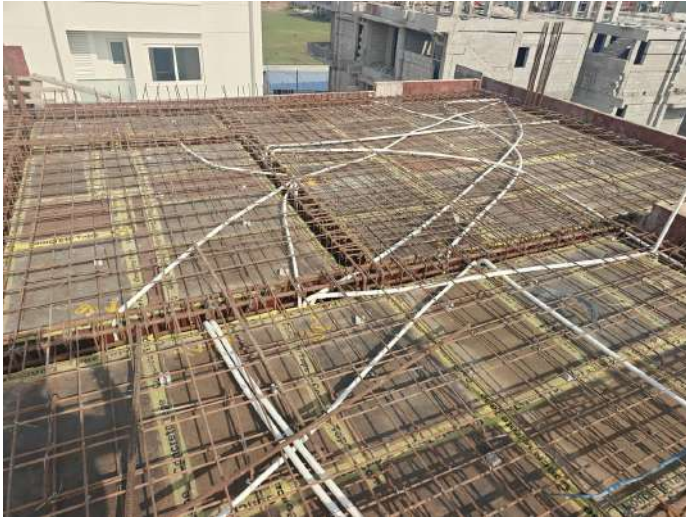
V97 - Staircase Headroom with Part Roof Slab & Beam - Electrical works
