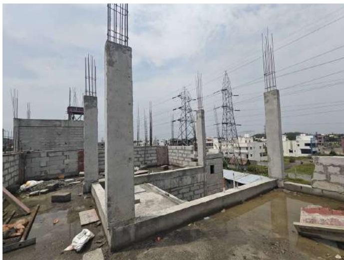
V81 - Stair Head Room Column Concreting
