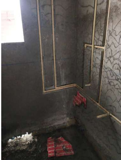
V38 - Internal Plumbing Core Cutting & Wall chasing
