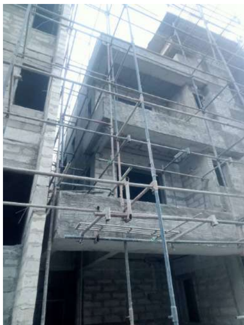
V43 - External Plastering
