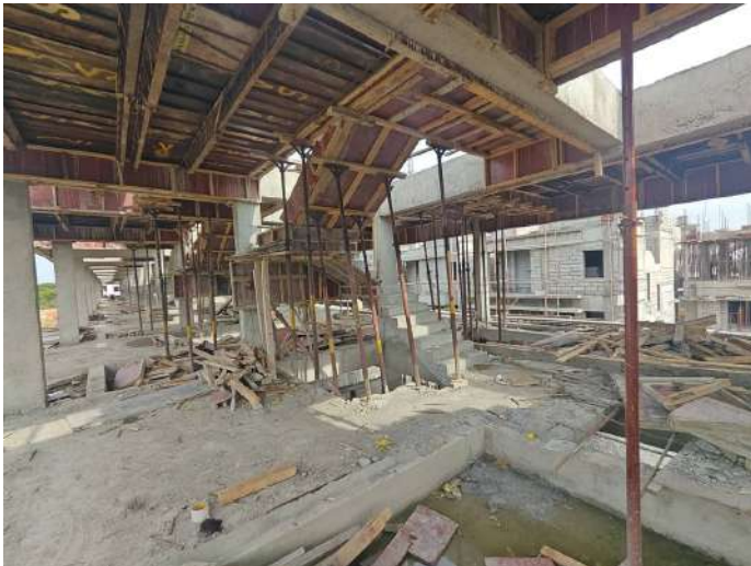
V84 - First Floor Column Concreting
