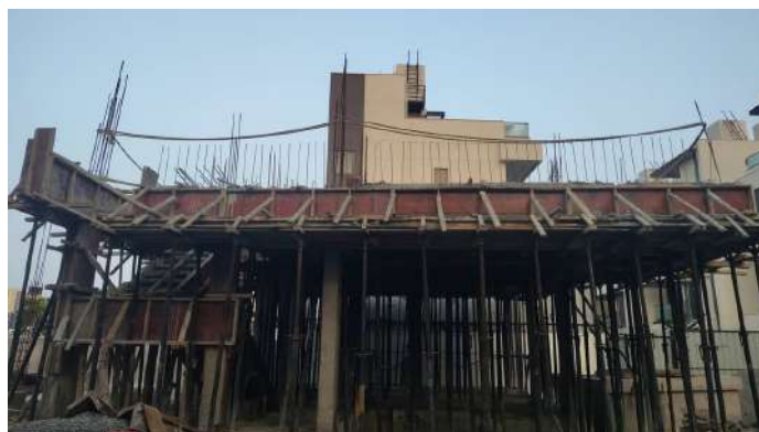
V123 - Completion of Ground Floor Roof Slab
