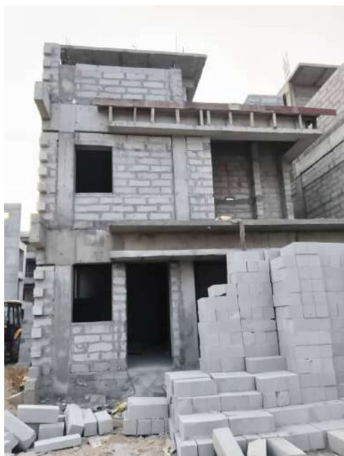
V53 - Instllation of Wall chasing & Electrical conduits
