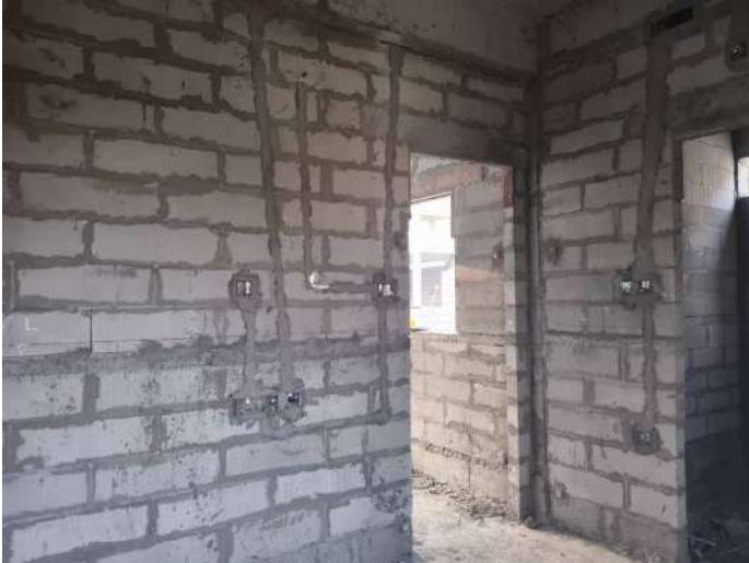
V31 - Instllation of Wall chasing & Electrical conduits
