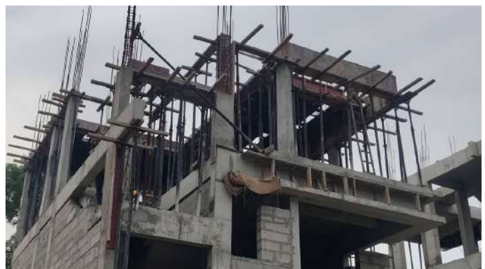
V109 - SF- Column Concreting
