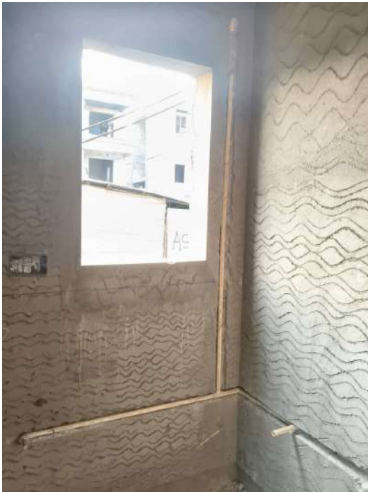
V29 - Instllation of Internal Plumbing
