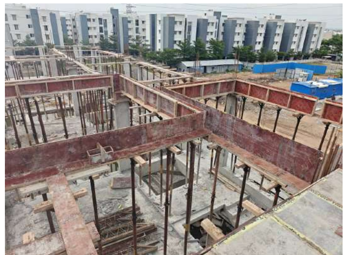
V86 - Stair Head Room Roof Slab & Beam - Electrical works
