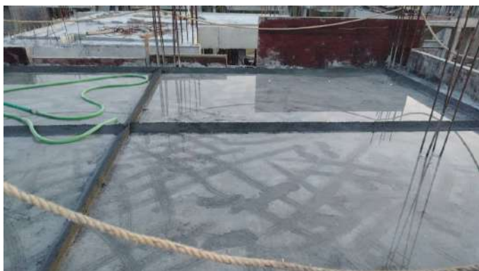
V119 - Completion of Staircase Headroom with Part roof slab
