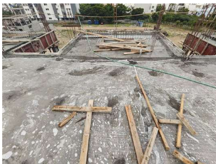
V95 - Completion of Staircase Headroom with Part roof slab
