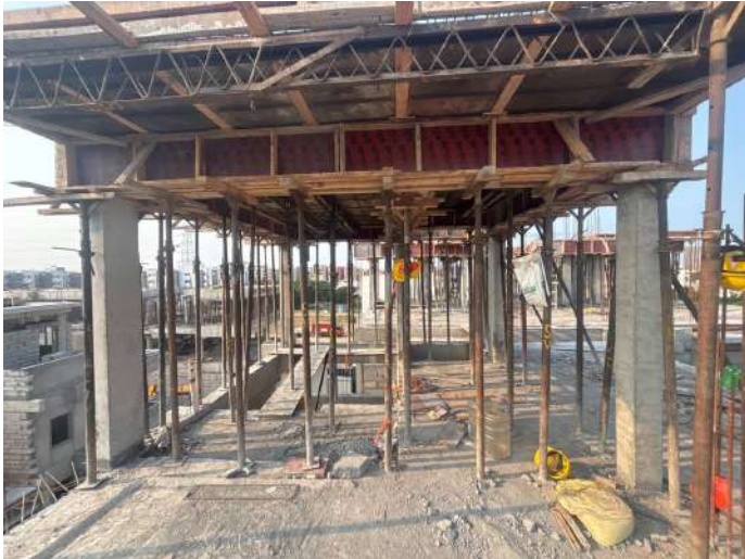
V106 - Stair Head Room Column Concreting
