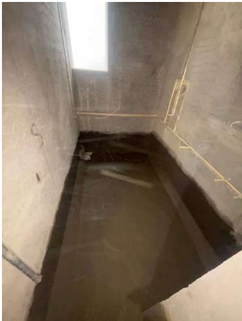
V70 - Toilet Waterproofing
