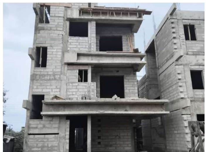
V30 - Completion of Blockwork
