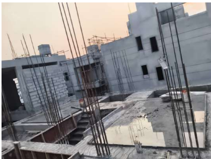
V35 - First Floor Roof Slab & Beam Concreting
