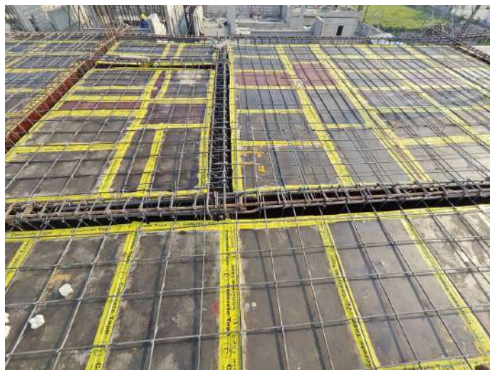
V85 - Stair Head Room Roof Slab & Beam - Shuttering, Reinforcement
