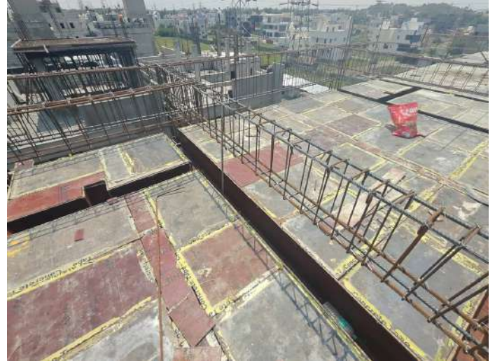
V86 - Stair Head Room Roof Slab & Beam - Shuttering, Reinforcement
