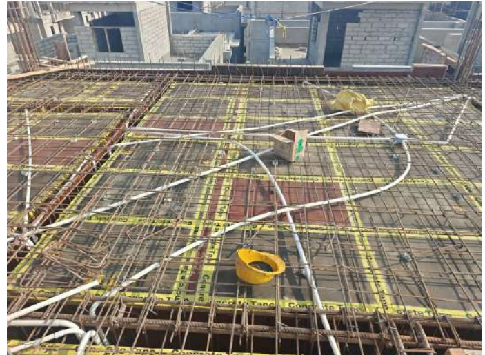
V96 - Staircase Headroom with Part Roof Slab & Beam - Electrical works
