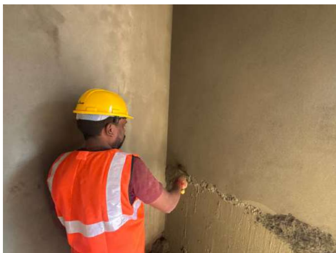
V107 - Internal Plastering
