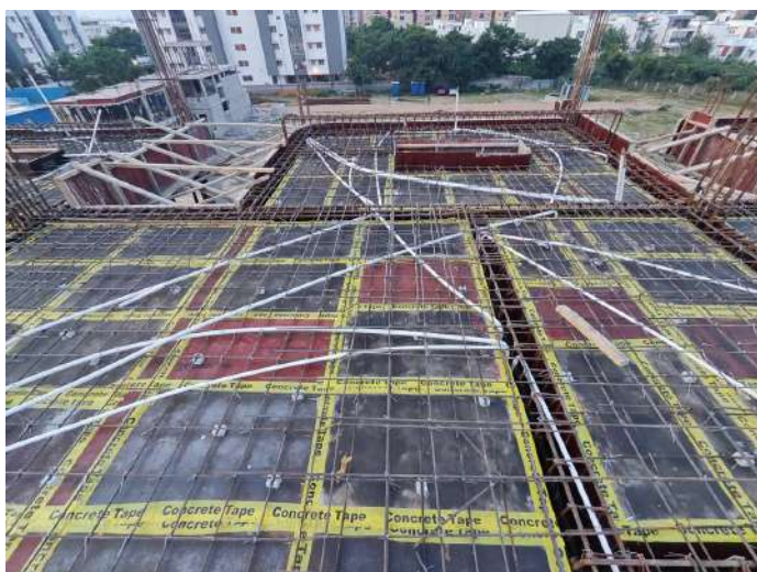
V92 - Stair Head Room Roof Slab & Beam - Electrical works
