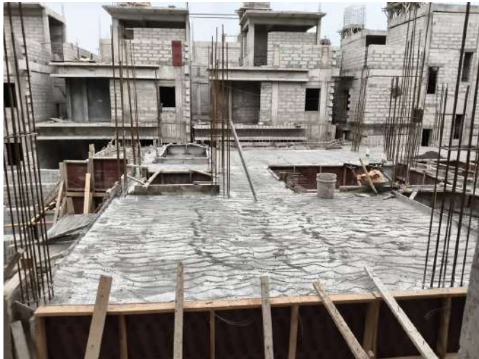
V35 - Completion of Ground Floor Roof Slab
