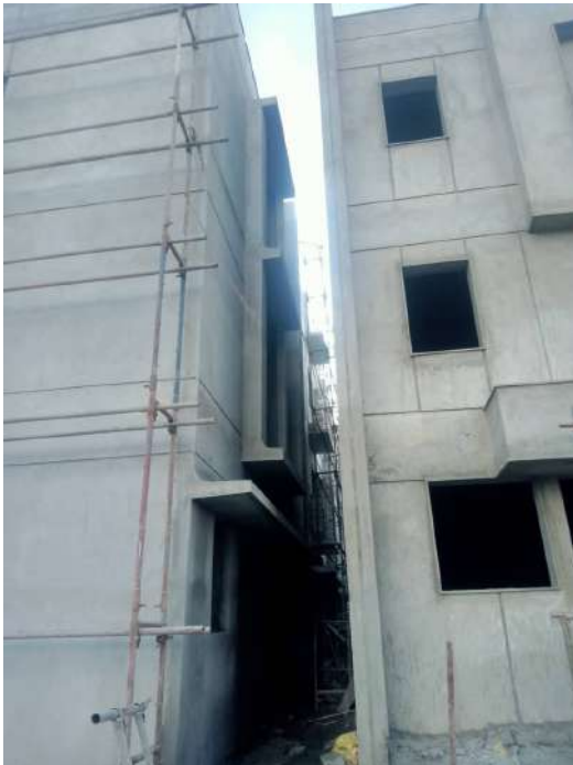
V43 - External Plastering
