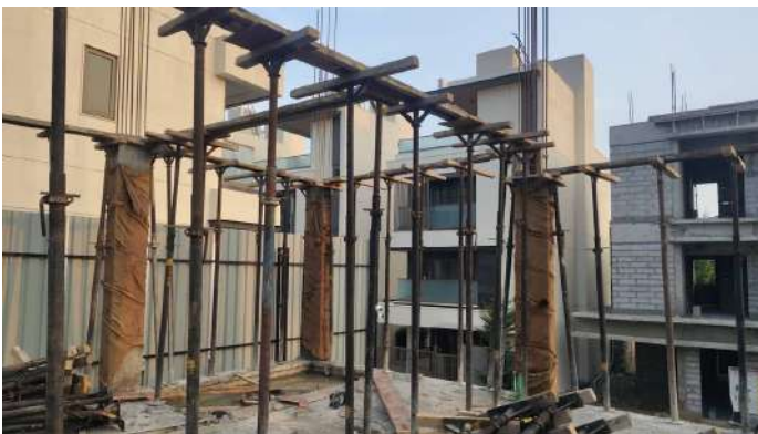
V123 - First Floor Roof Slab & Beam - Shuttering, Reinforcement
