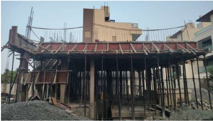
V123 - Ground Floor Roof Slab & Beam Concreting
