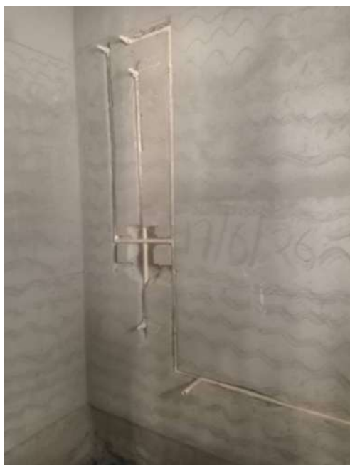
V47 - Internal Plumbing Core Cutting & Wall chasing
