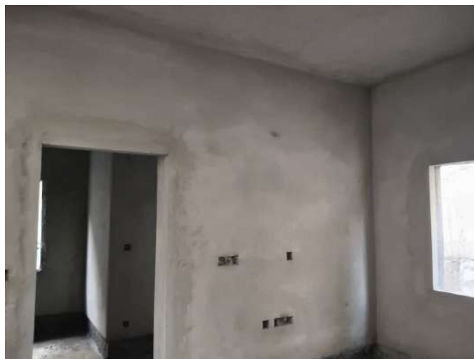
V31 - Internal Plastering
