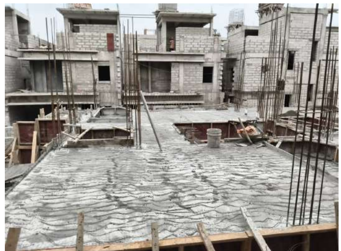
V35 - Ground Floor Roof Slab & Beam Concreting
