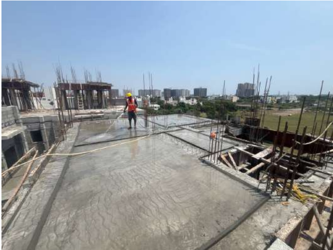
V103 - SF- Roof Slab & Beam - Shuttering, Reinforcement
