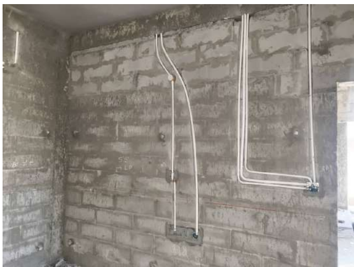
V56 - Instllation of Wall chasing & Electrical conduits
