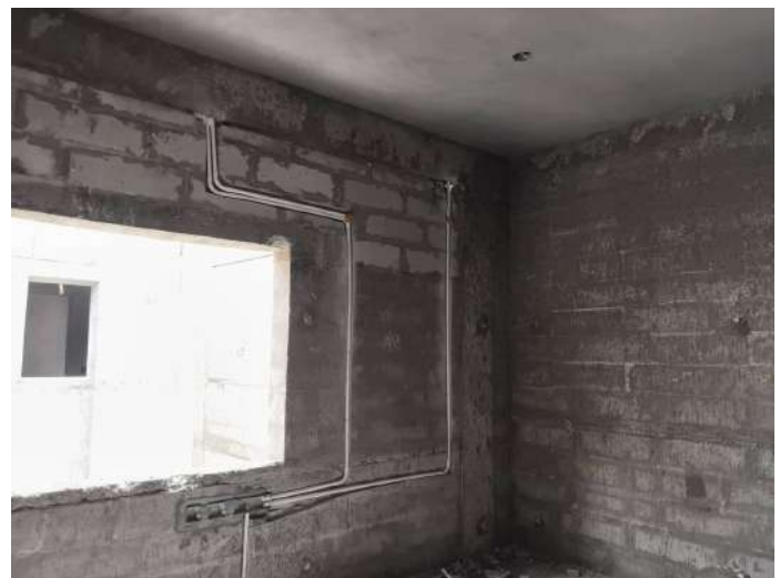
V56 - Completion of Blockwork
