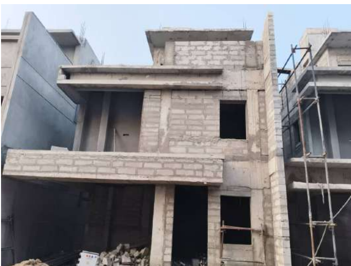
V48 - Internal Plastering
