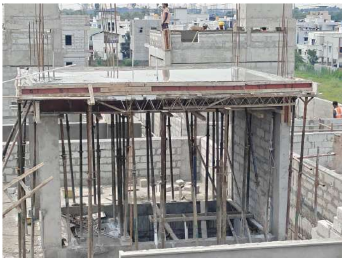
V80 - Stair Head Room Roof Slab & Beam Concreting
