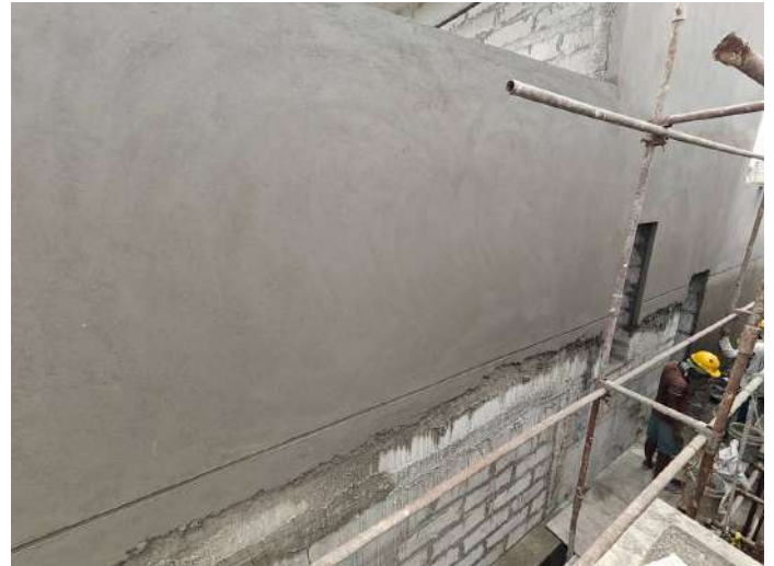
V74 - External Plastering
