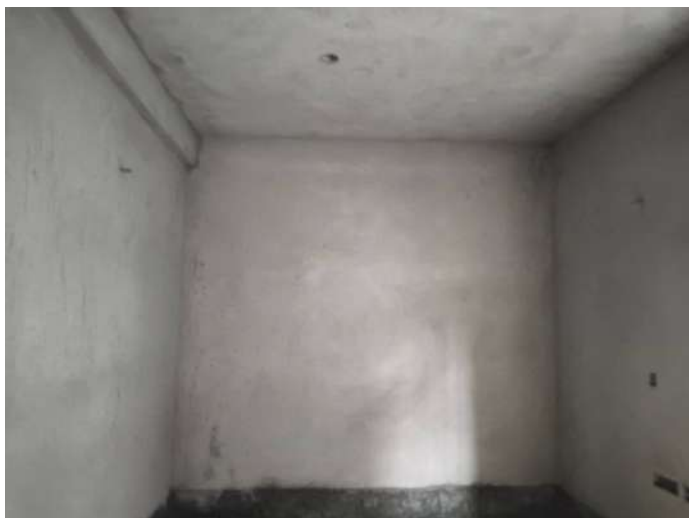
V31 - Internal Plastering
