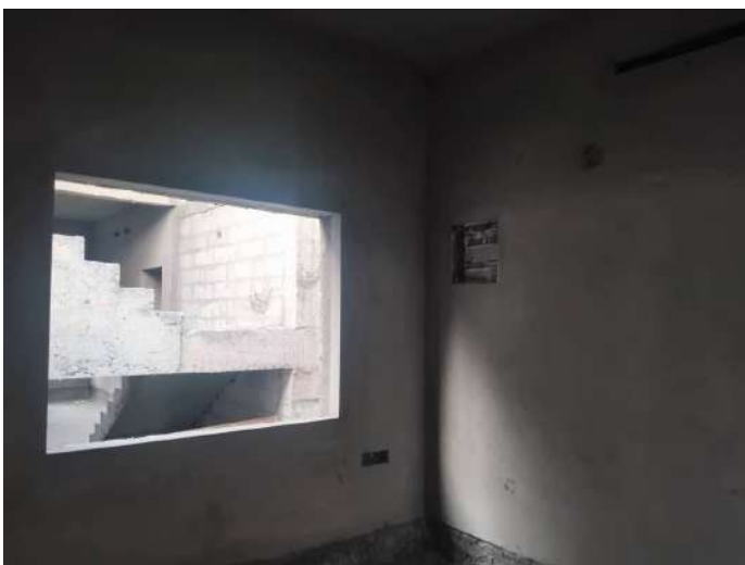
V31 - Internal Plastering
