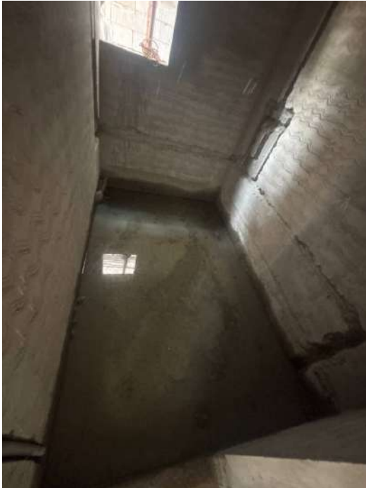
V69 - Toilet Waterproofing
