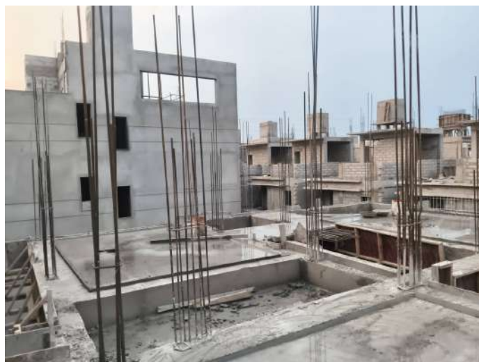
V35 - First Floor Roof Slab & Beam Concreting
