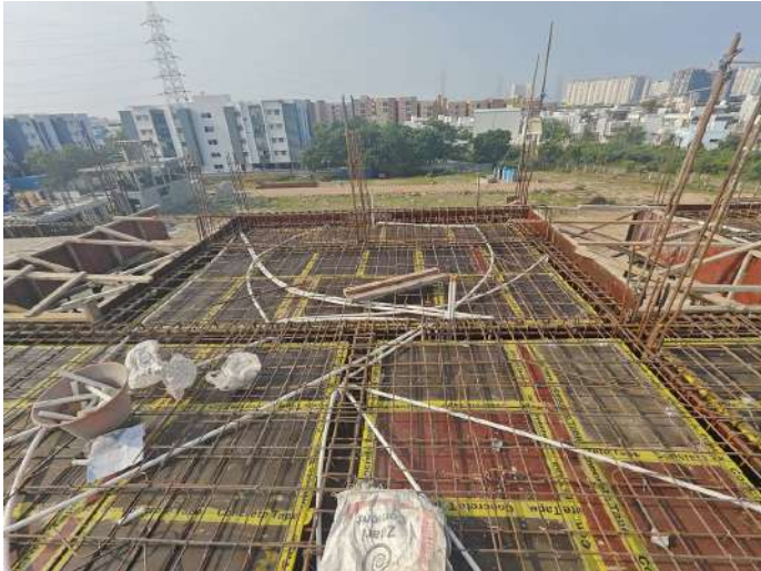
V94 - Stair Headroom with Part Roof Slab & Beam - Shuttering, Reinforcement
