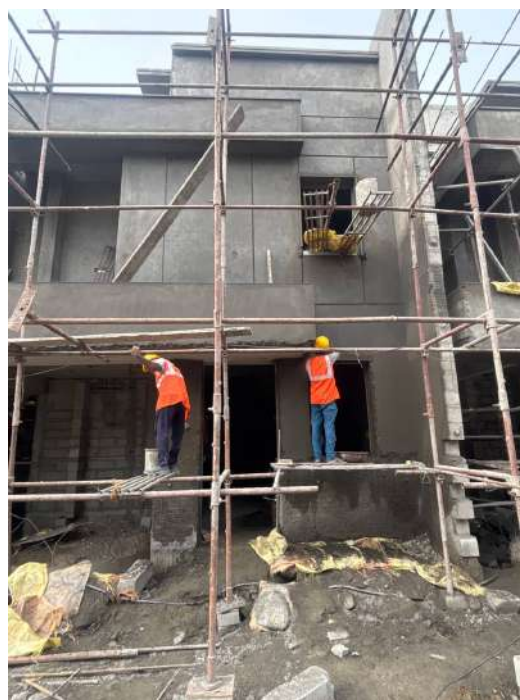
V65 - External Plastering
