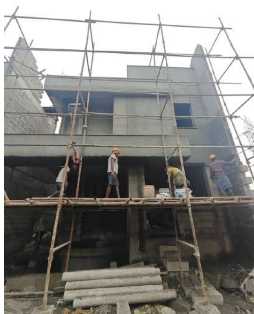
V81 - External Plastering
