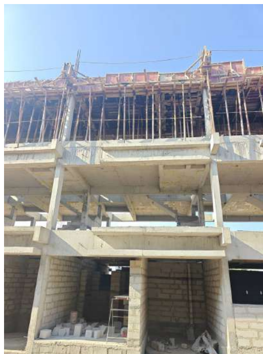
V91 - Stair Head Room Roof Slab & Beam Concreting
