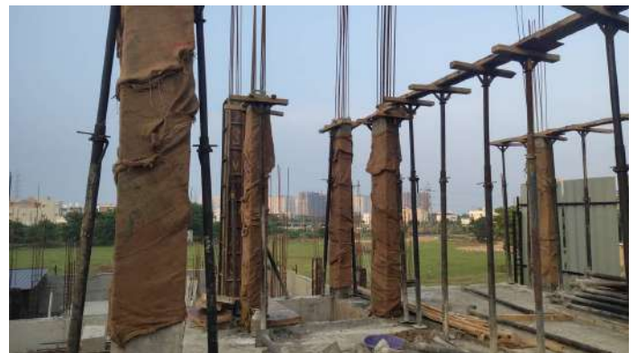
V123 - First Floor Column Concreting
