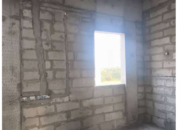
V31 - Instllation of Wall chasing & Electrical conduits
