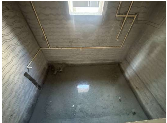
V70 - Toilet Waterproofing
