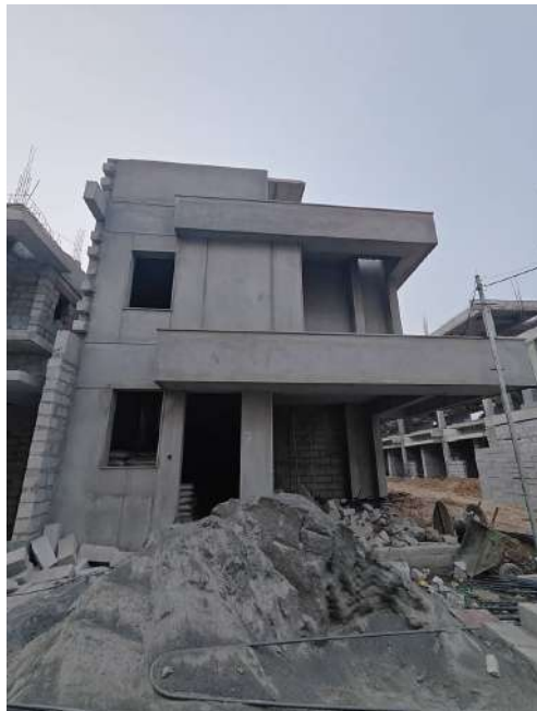
V73 - External Plastering
