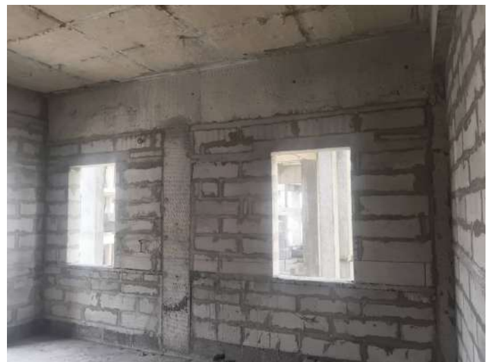
V27 - Completion of Blockwork
