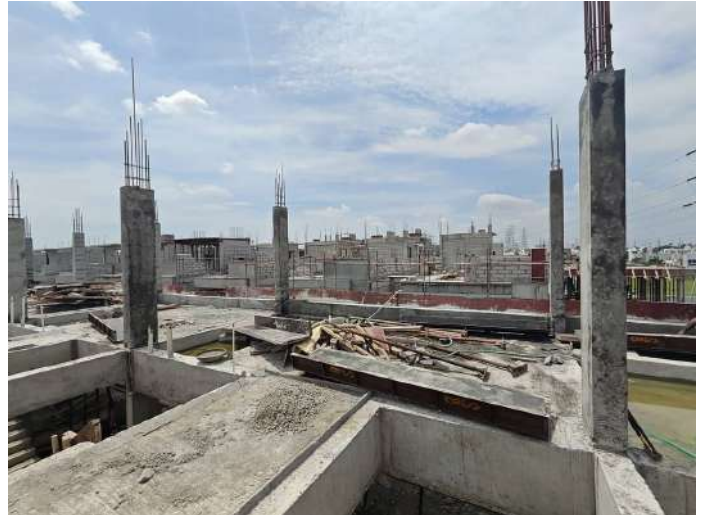
V85 - Stair Head Room Column Concreting
