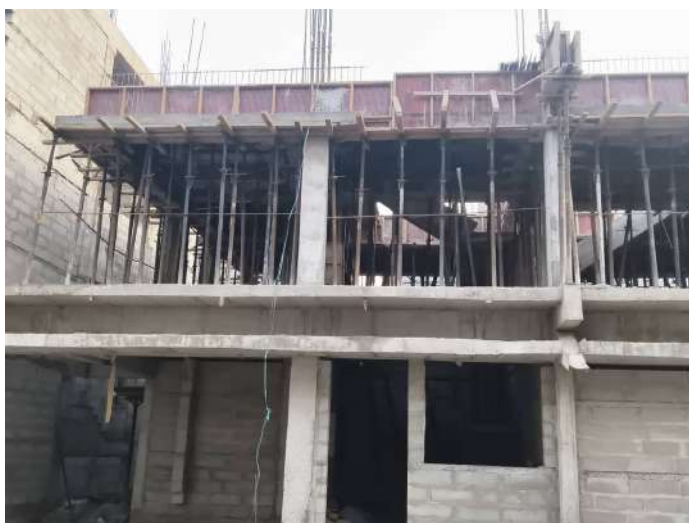
V34 - Completion of First Floor Roof Slab
