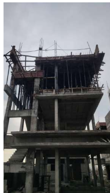
V113 - Completion of Second Floor Roof Slab
