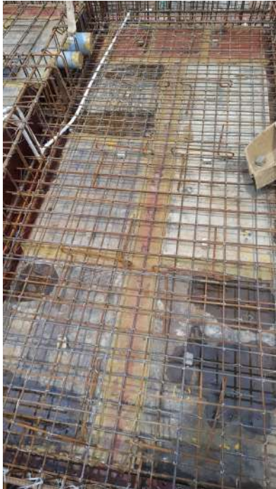
V123 - Ground Floor Roof Slab & Beam - Shuttering, Reinforcement
