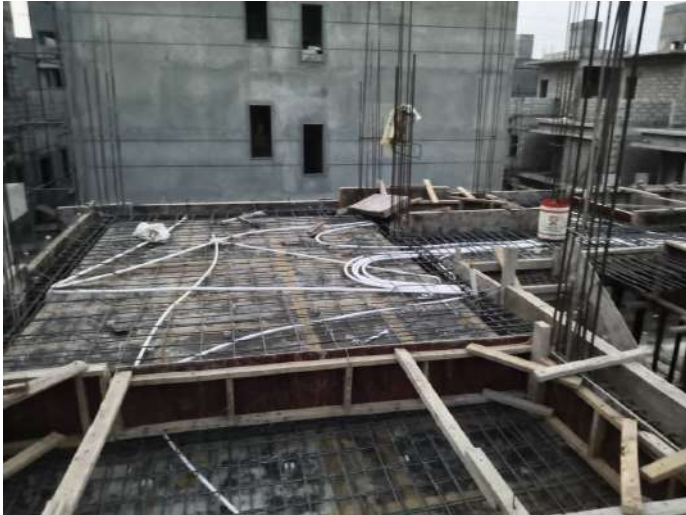
V35 - First Floor Roof Slab & Beam - Electrical works
