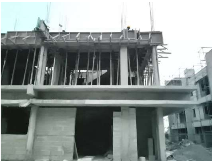
V35 - First Floor Roof Slab & Beam - Shuttering, Reinforcement
