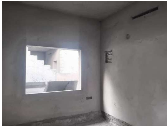
V31 - Internal Plastering
