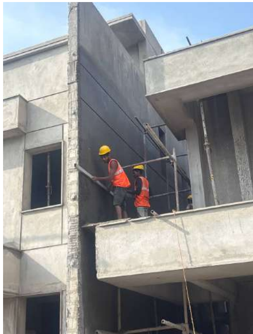
V65 - External Plastering
