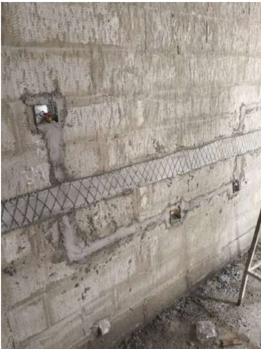
V31 - Instllation of Wall chasing & Electrical conduits
