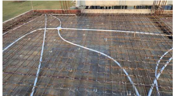
V119 - Stair Head Room with Part Roof Slab & Beam - Electrical works
