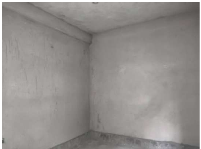
V31 - Internal Plastering
