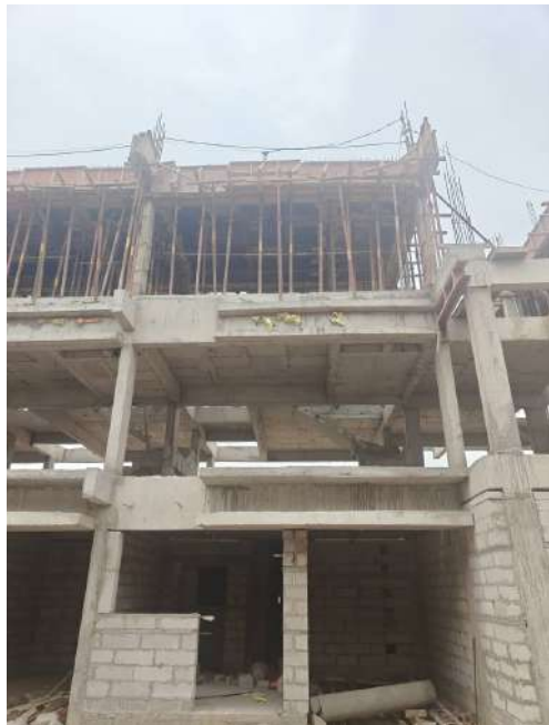
V96 - Completion of Staircase Headroom with Part roof slab
