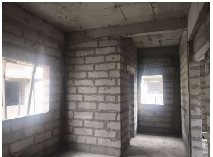
V36 - Completion of Blockwork
