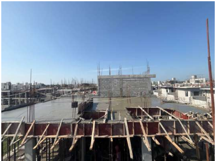
V107 - Completion of Second Floor Roof Slab
