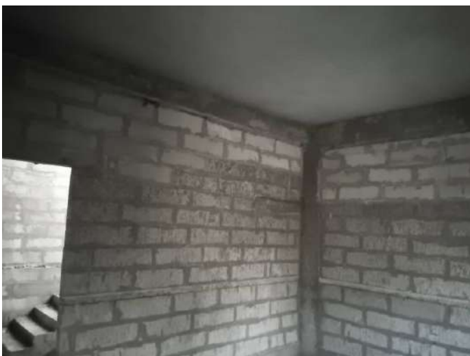
V58 - Completion of Blockwork
