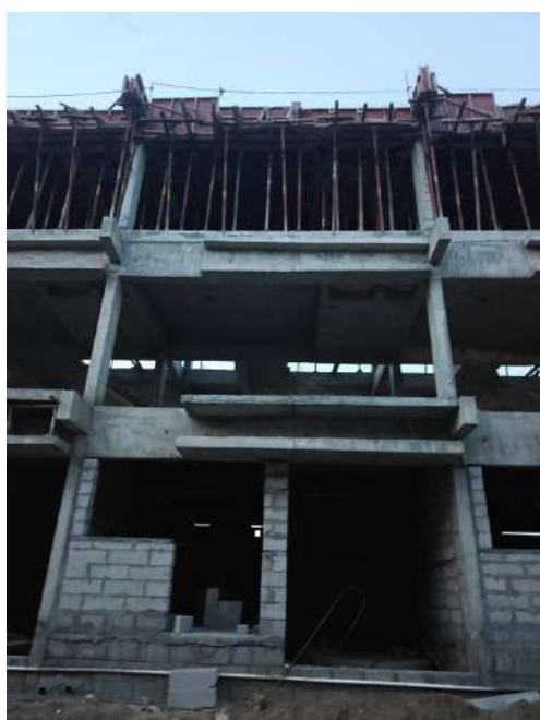
V86 - Stair Head Room Roof Slab & Beam - Shuttering, Reinforcement
