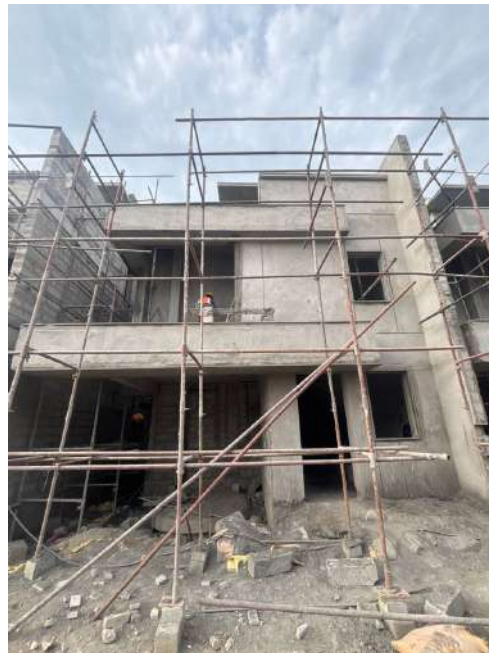
V65 - External Plastering
