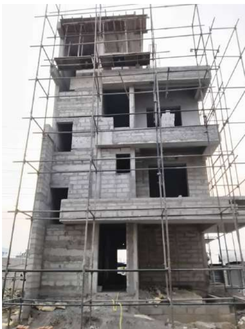
V46 - Instllation of Wall chasing & Electrical conduits
