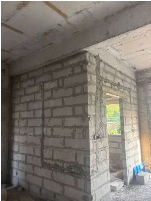
V23 - Completion of Blockwork
