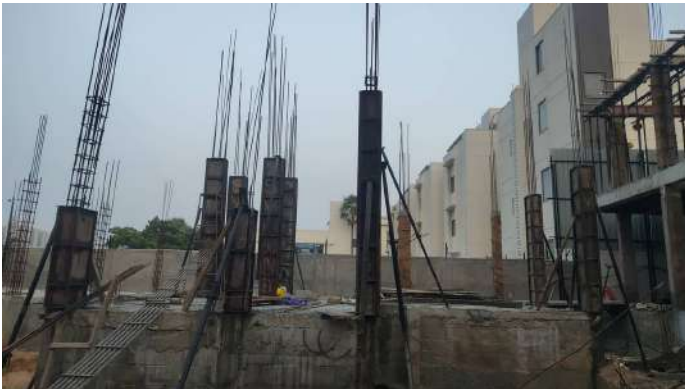
V122 - Ground Floor Column Concreting
