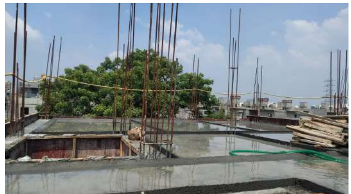
V109 - Completion of Second Floor Roof Slab
