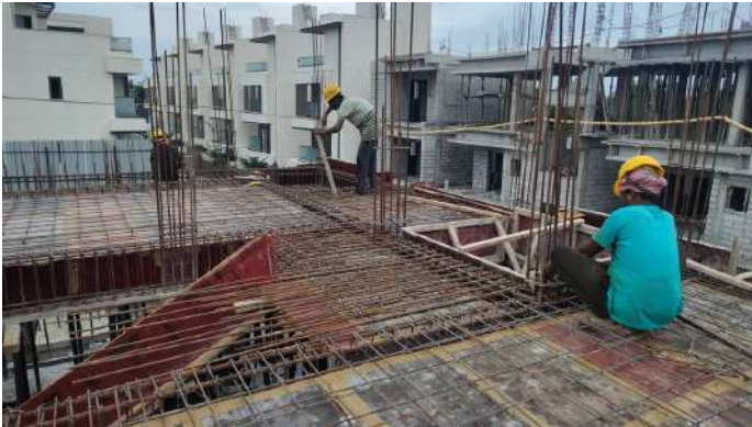
V117 - First Floor Roof Slab & Beam - Shuttering, Reinforcement
