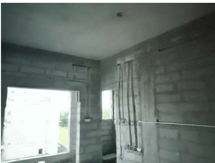
V30 - Completion of Blockwork
