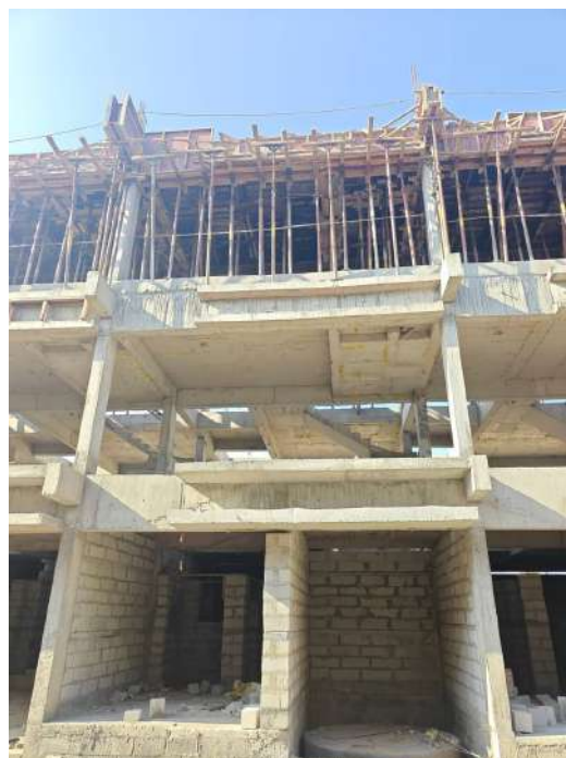
V90 - Stair Head Room Roof Slab & Beam Concreting
