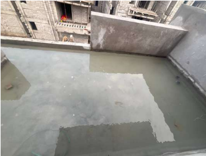
V71 - Terrace Waterproofing
