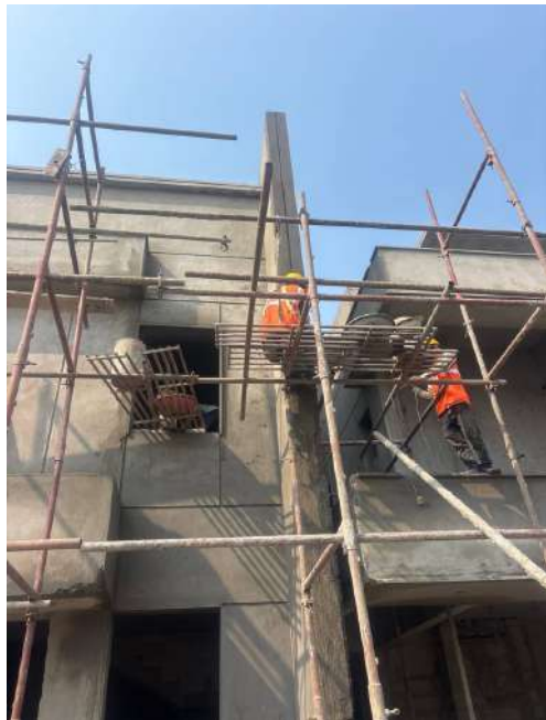
V64 - External Plastering
