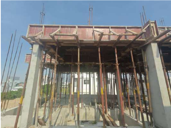
V98 - Staircase Headroom Roof Slab & Beam - Shuttering, Reinforcement
