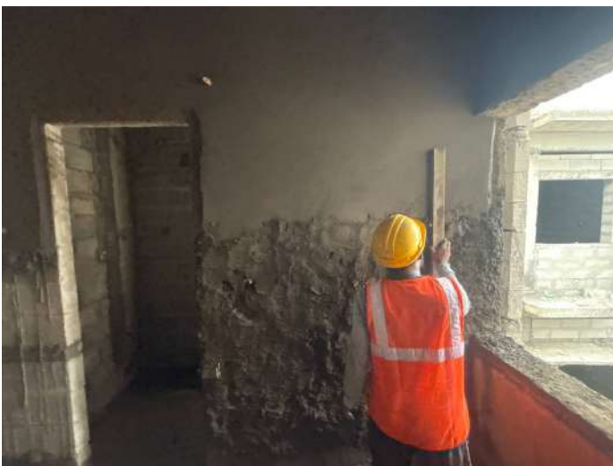
V106 - Internal Plastering
