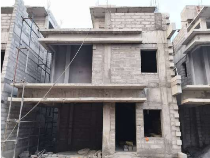
V49 - Instllation of Wall chasing & Electrical conduits
