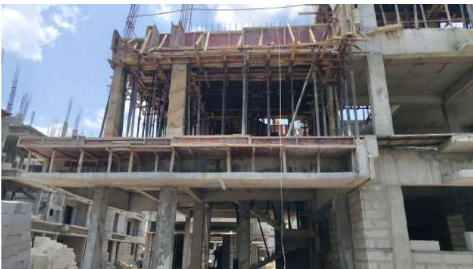
V117 - Completion of First Floor Roof Slab
