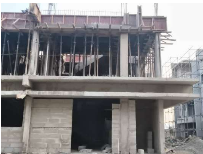
V35 - Completion of First Floor Roof Slab
