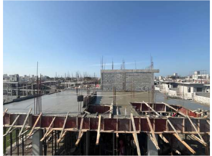
V107 - SF- Roof Slab & Beam Concreting
