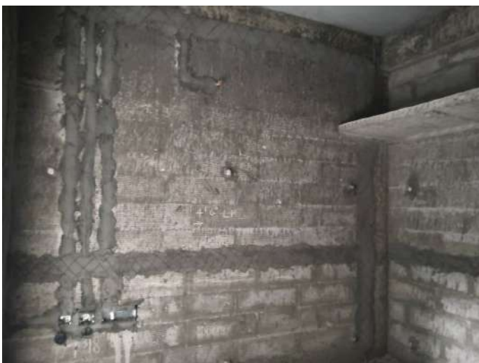
V55 - Instllation of Wall chasing & Electrical conduits
