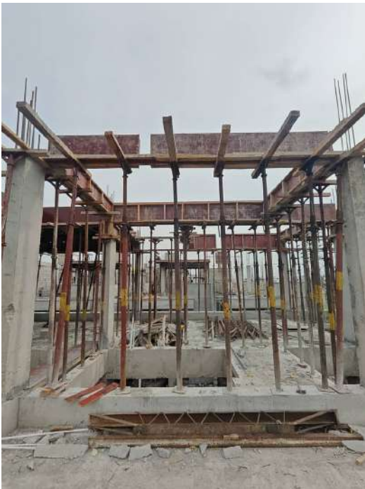
V86 - Stair Head Room Roof Slab & Beam - Electrical works
