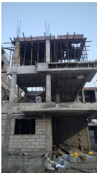
V115 - Staircase Headroom with Part Roof Slab & Beam - Shuttering, Reinforcement
