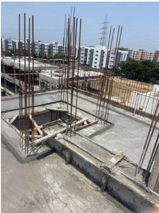
V105 - Stair Head Room Roof Slab & Beam Concreting
