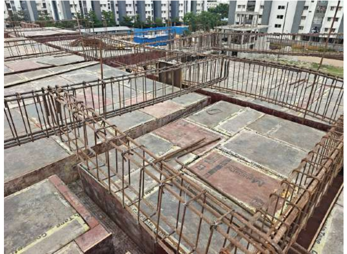
V92 - Stair Head Room Roof Slab & Beam - Shuttering, Reinforcement
