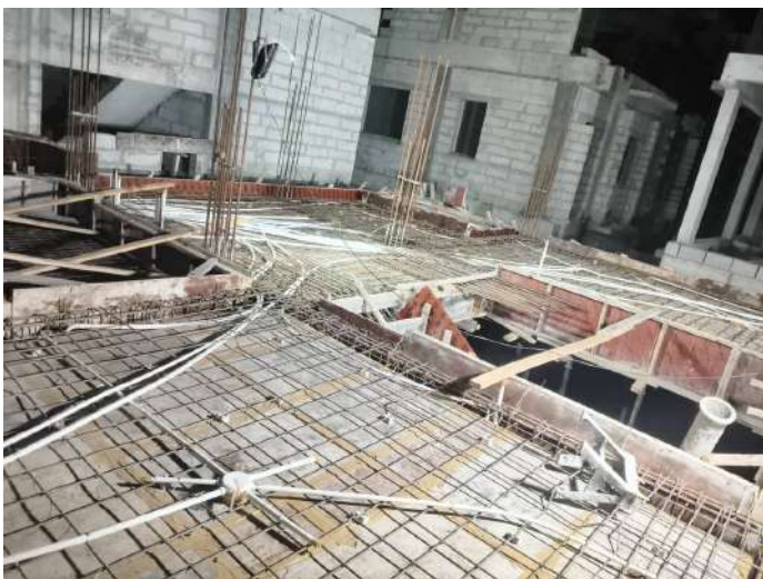
V34 - Ground Floor Roof Slab & Beam - Electrical works
