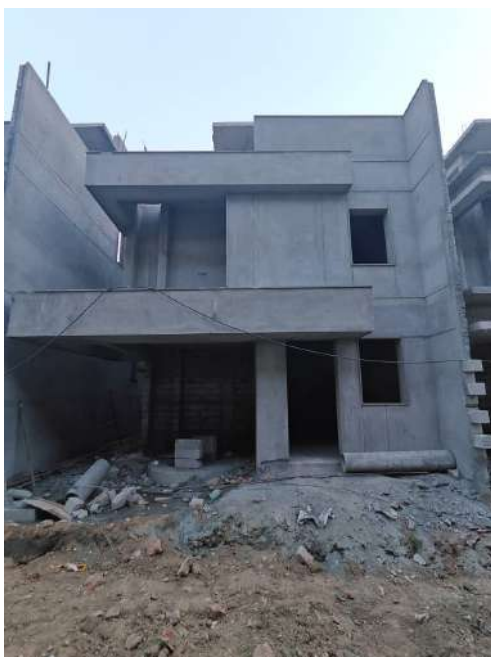
V75 - External Plastering
