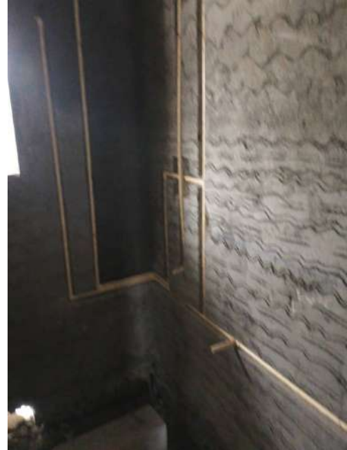
V37 - Internal Plumbing Core Cutting & Wall chasing
