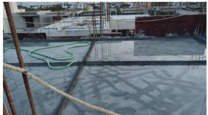
V119 - Stair Head Room with Part Roof Slab & Beam Concreting
