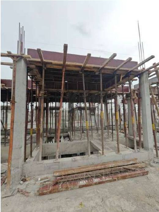
V87 - Stair Head Room Roof Slab & Beam - Shuttering, Reinforcement
