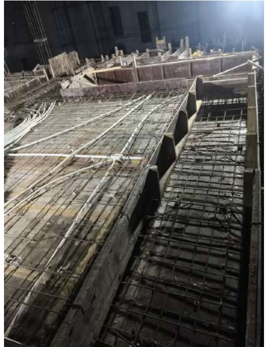
V35 - Ground Floor Roof Slab & Beam - Shuttering, Reinforcement
