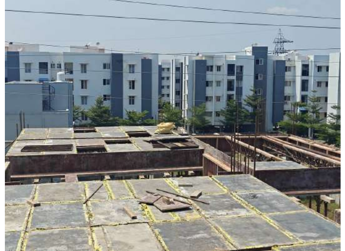
V83 - Stair Head Room Roof Slab & Beam - Shuttering, Reinforcement
