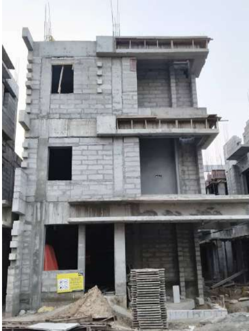
V32 - Internal Plastering
