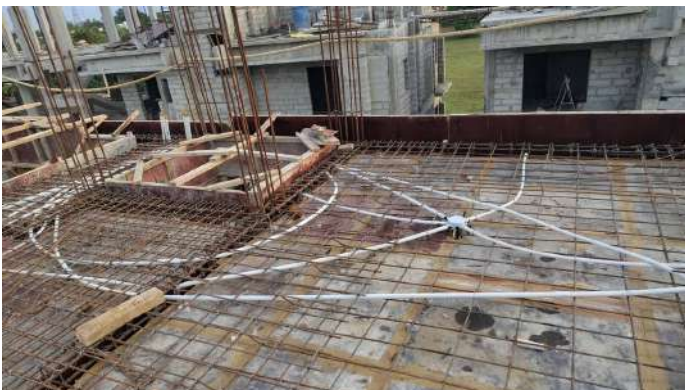
V109 - SF- Roof Slab & Beam - Electrical works
