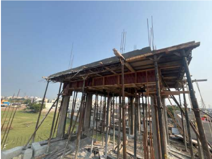
V103 - Stair Head Room Roof Slab & Beam Concreting
