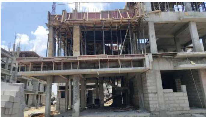
V117 - First Floor Roof Slab & Beam Concreting
