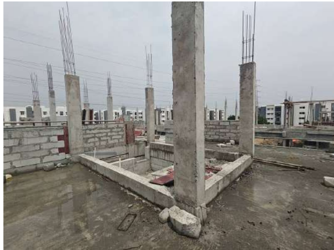
V80 - Stair Head Room Column Concreting
