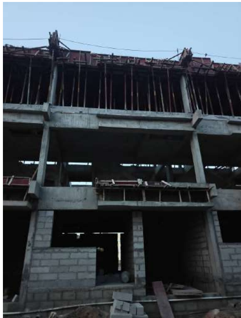
V85 - Stair Head Room Roof Slab & Beam - Shuttering, Reinforcement
