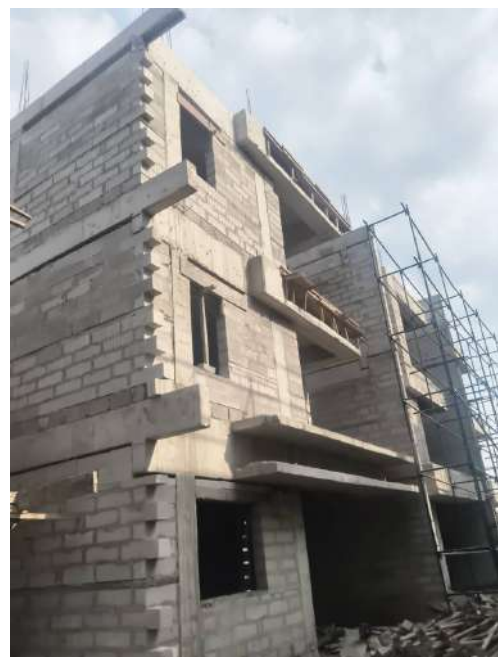
V36 - Completion of Blockwork
