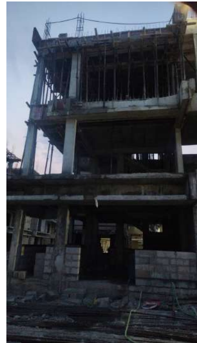
V117 - SF- Roof Slab & Beam Concreting
