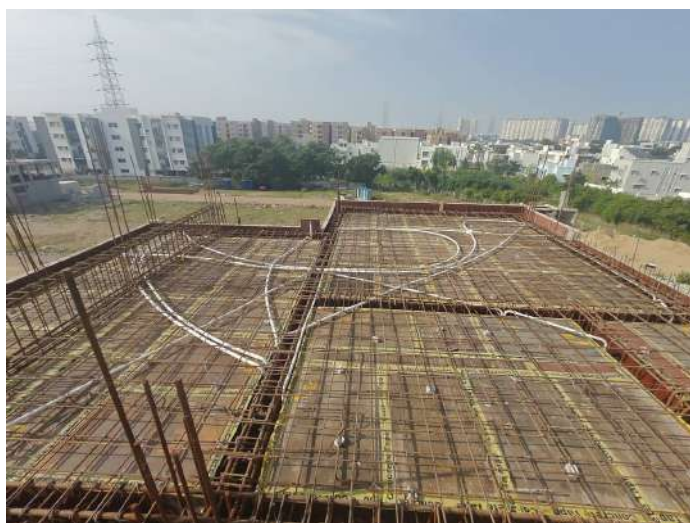
V98 - Staircase Headroom Roof Slab & Beam - Electrical works
