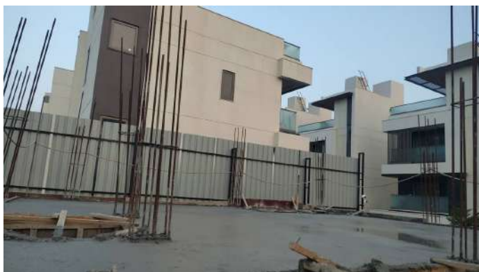
V123 - Completion of Ground Floor Roof Slab
