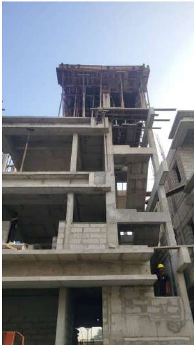
V26 - Stair Head Room Roof Slab & Beam - Shuttering, Reinforcement
