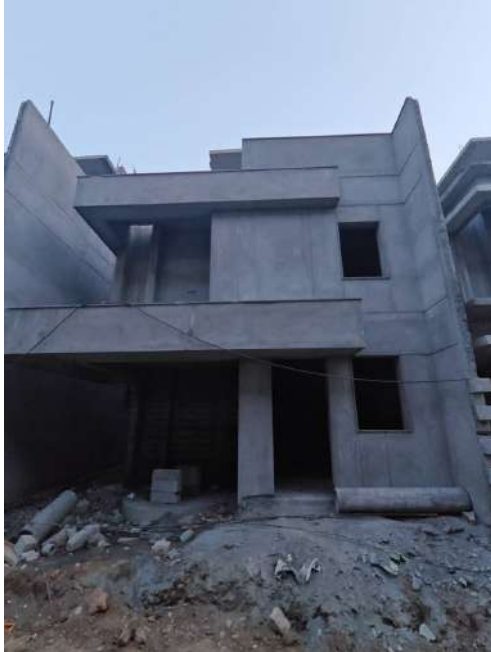
V76 - External Plastering
