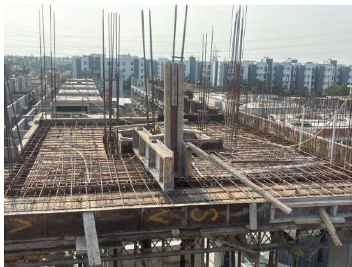
V105 - Stair Head Room Roof Slab & Beam - Shuttering, Reinforcement
