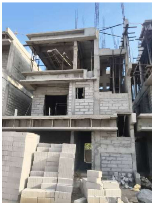
V24 - SF- Roof Slab & Beam Concreting
