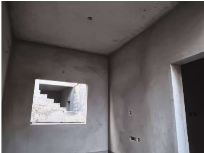
V52 - Internal Plastering
