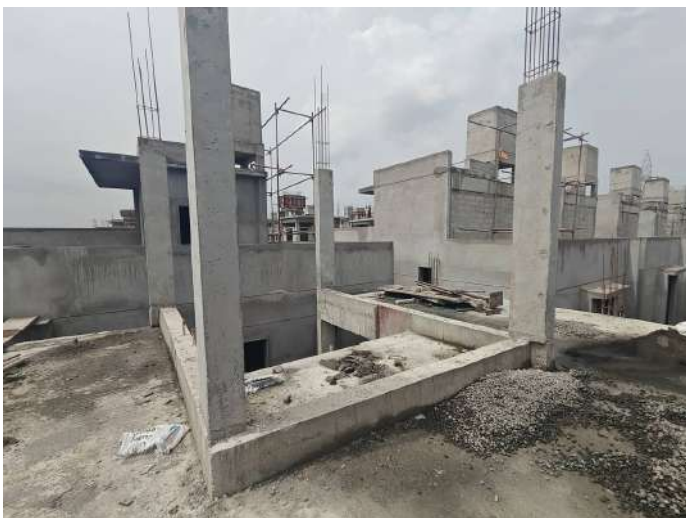
V72 - Stair Head Room Column Concreting
