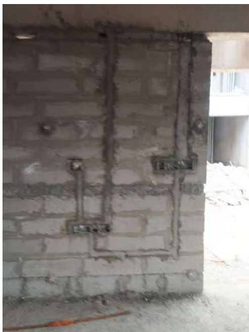
V104 - Instllation of Wall chasing & Electrical conduits
