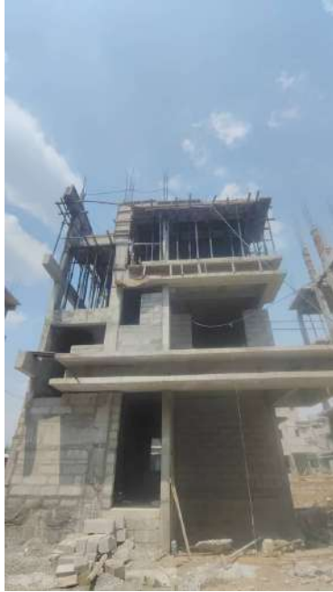
V109 - SF- Roof Slab & Beam Concreting
