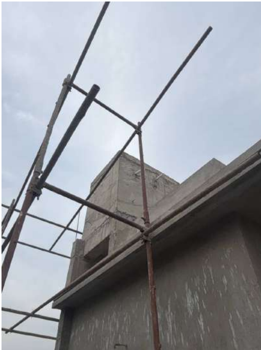
V70 - OHT Cover Slab Concreting
