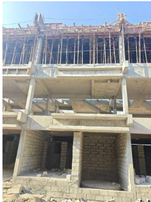
V90- Completion of Staircase Headroom & Part Roof Slab
