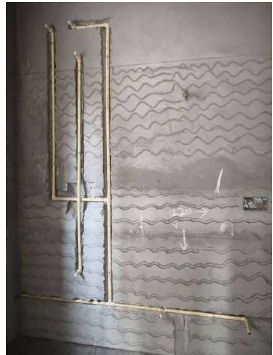
V29 - Instllation of Internal Plumbing
