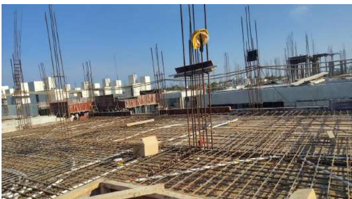
V113 - SF- Roof Slab & Beam - Shuttering, Reinforcement
