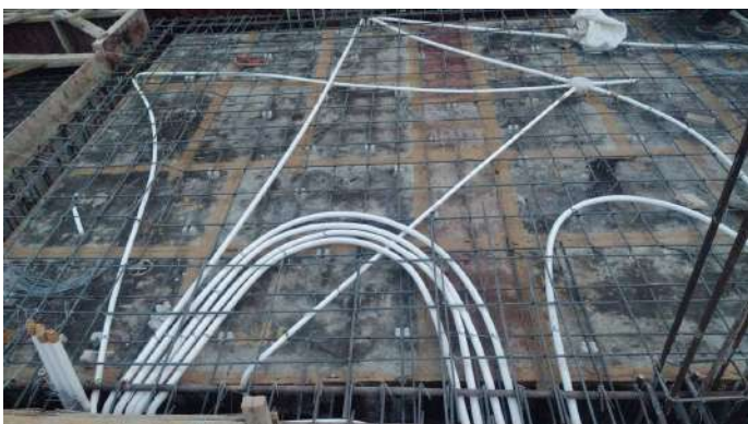
V117 - SF- Roof Slab & Beam - Electrical works
