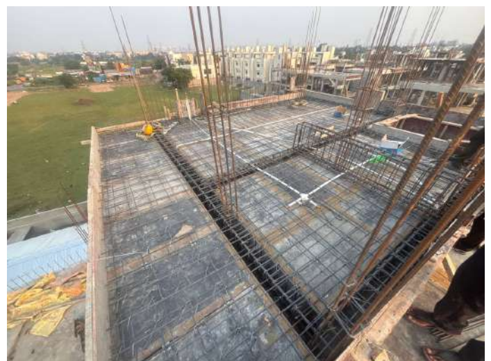
V103 - Stair Head Room Roof Slab & Beam - Shuttering, Reinforcement
