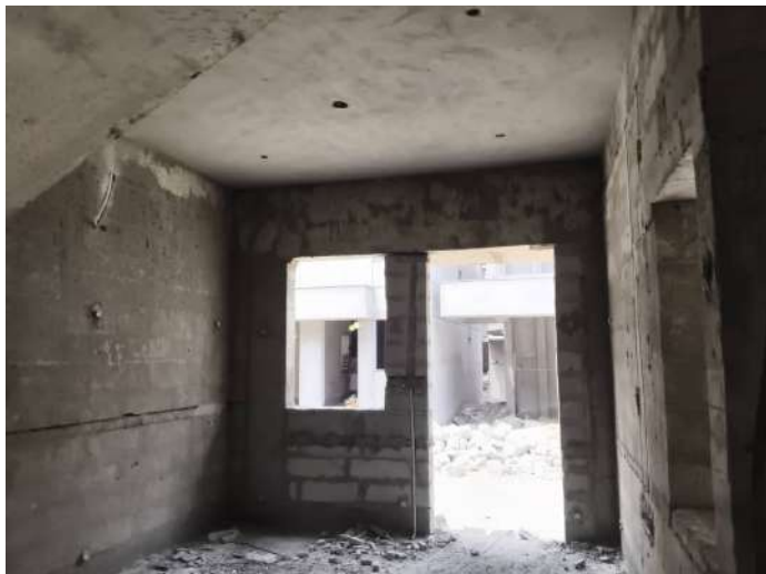
V56 - Completion of Blockwork
