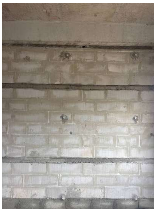
V108 - Completion of Blockwork
