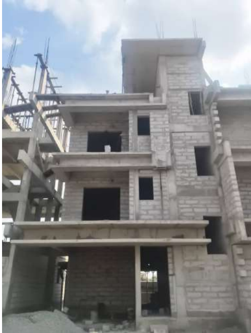
V27 - Completion of Blockwork
