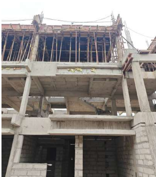
V96 - Completion of Staircase Headroom with Part roof slab
