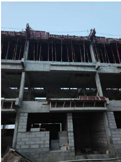
V84 - Stair Head Room Roof Slab & Beam - Shuttering, Reinforcement
