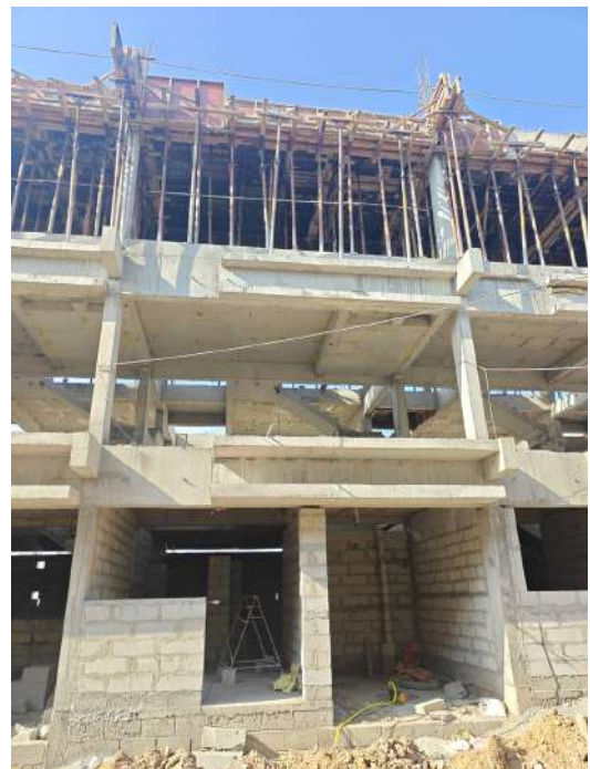
V93 - Stair Head Room Roof Slab & Beam Concreting
