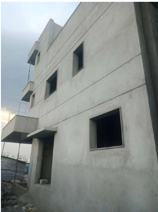
V45 - External Plastering
