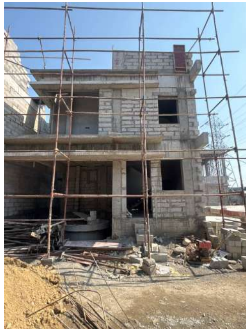
V81 - Completion of Blockwork
