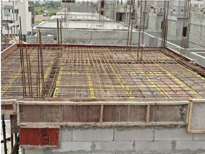
V79 - Stair Head Room Roof Slab & Beam - Shuttering, Reinforcement
