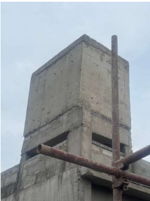
V65 - OHT Cover Slab Concreting
