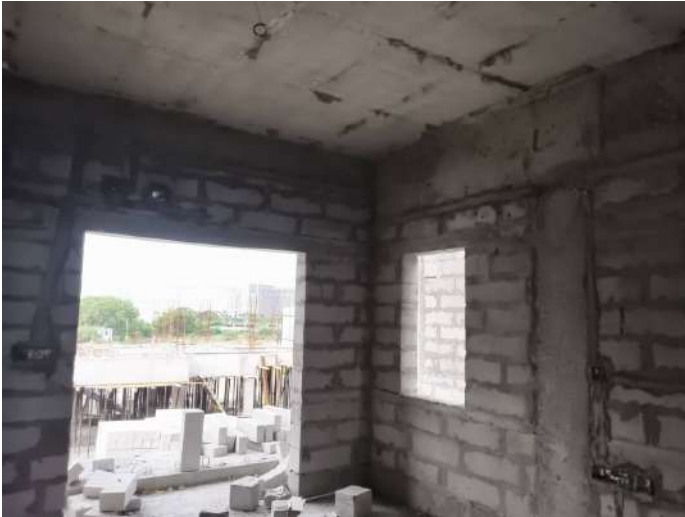
V23 - Completion of Blockwork
