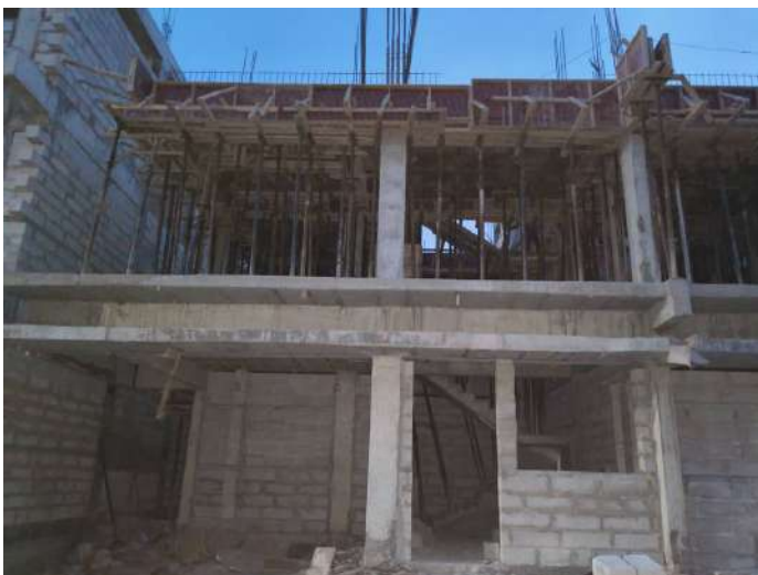
V34 - First Floor Roof Slab & Beam - Shuttering, Reinforcement
