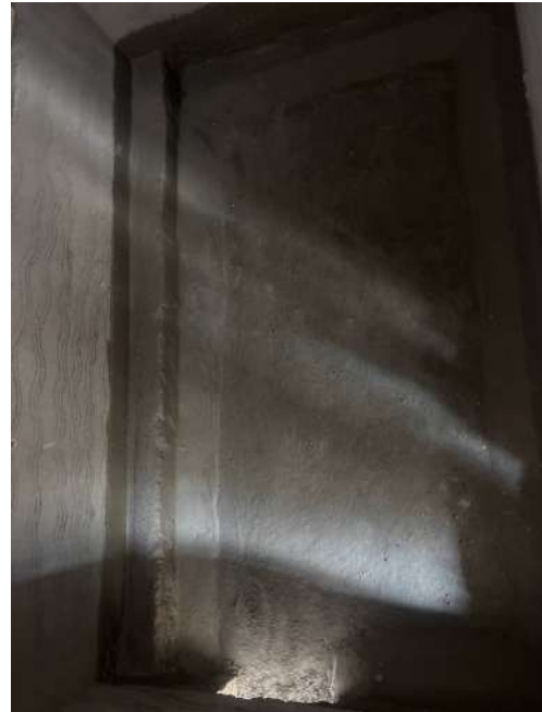
V71 - Toilet Waterproofing
