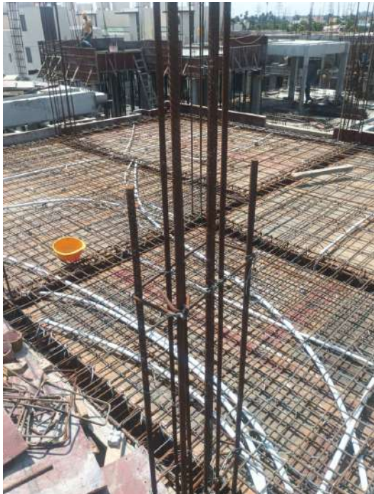
V113 - SF- Roof Slab & Beam - Electrical works
