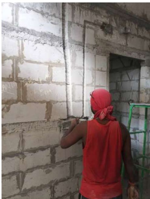
V97 - Instllation of Wall chasing & Electrical conduits
