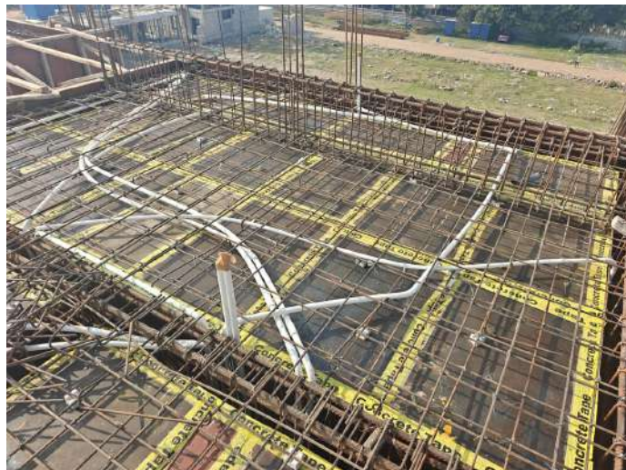
V95 - Staircase Headroom with Part Roof Slab - Electrical works
