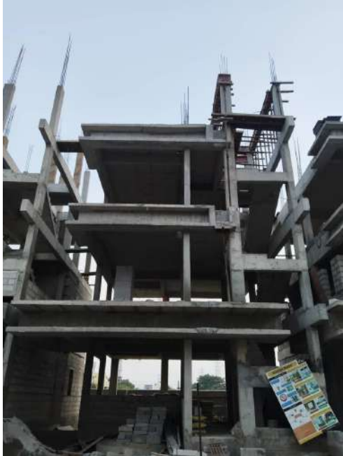
V25 - Stair Head Room Roof Slab & Beam - Shuttering, Reinforcement
