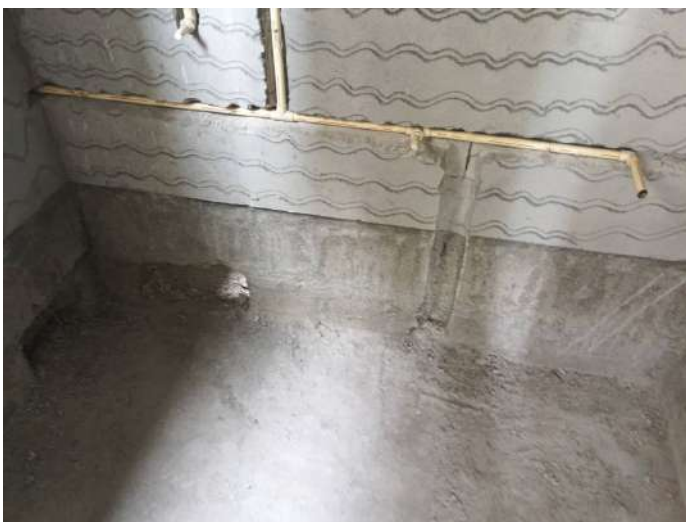
V29 - Internal Plumbing Core Cutting & Wall chasing
