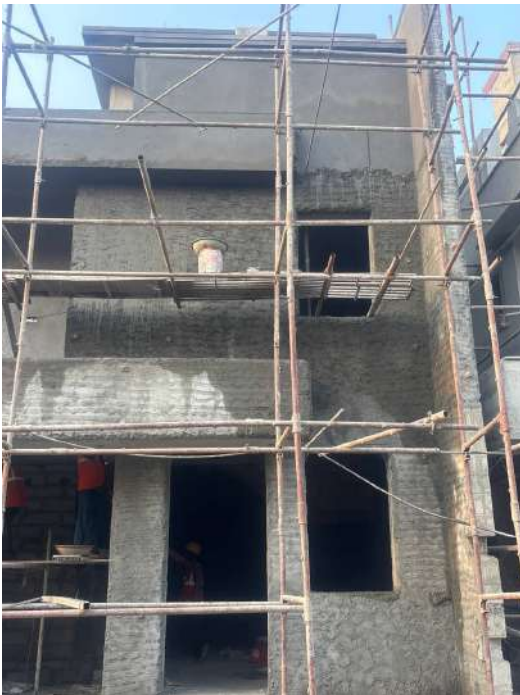
V66 - External Plastering
