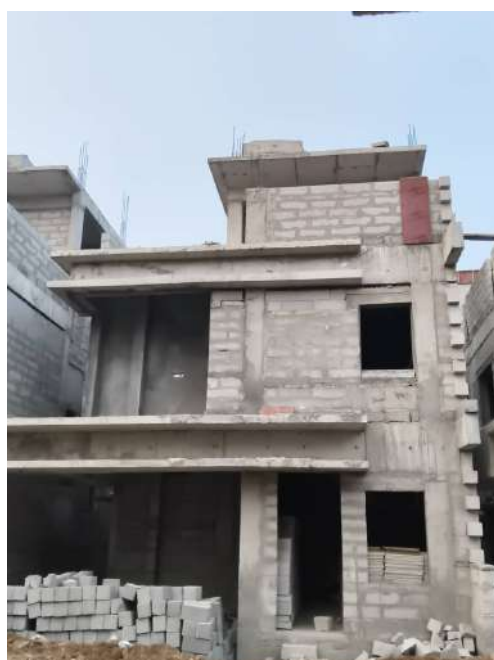
V51 - Installation of Wall chasing & Electrical conduits
