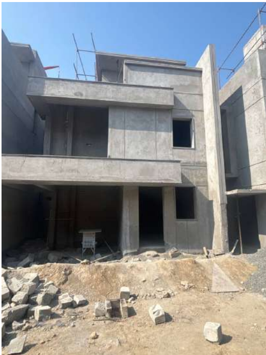
V70 - External Plastering
