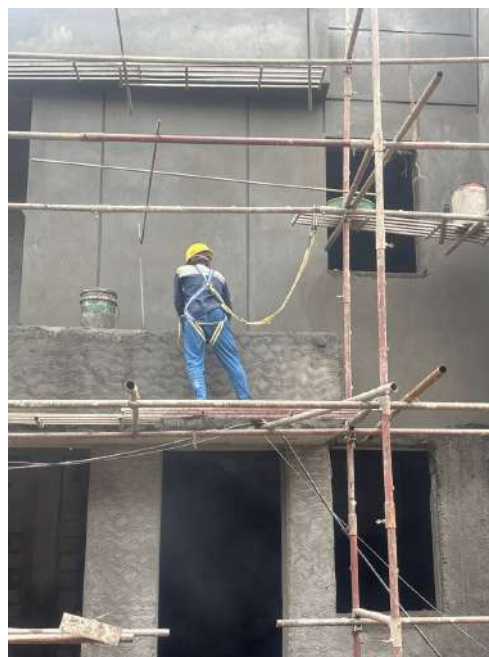
V68 - External Plastering
