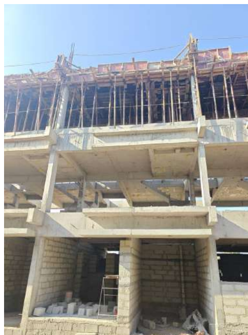
V91 - Completion of Staircase Headroom & Part Roof Slab
