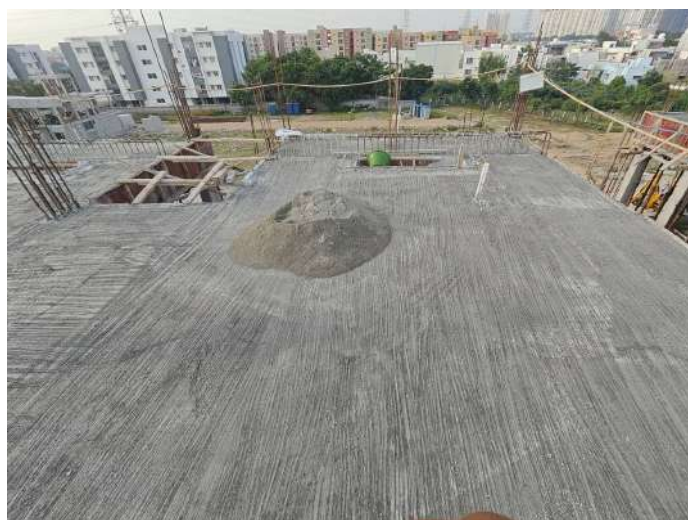
V96 - Staircase Headroom with Part Roof Slab & Beam Concreting
