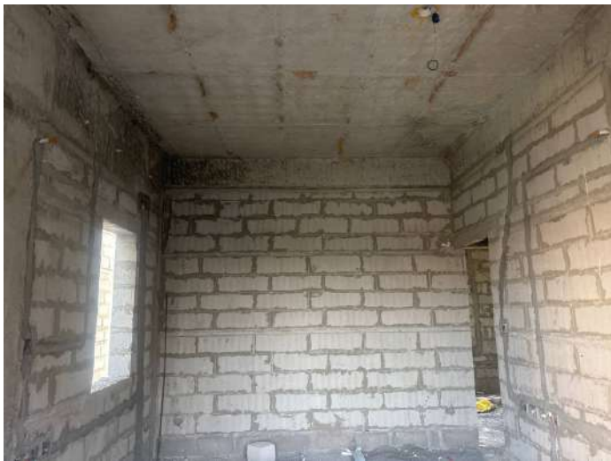
V23 - Completion of Blockwork
