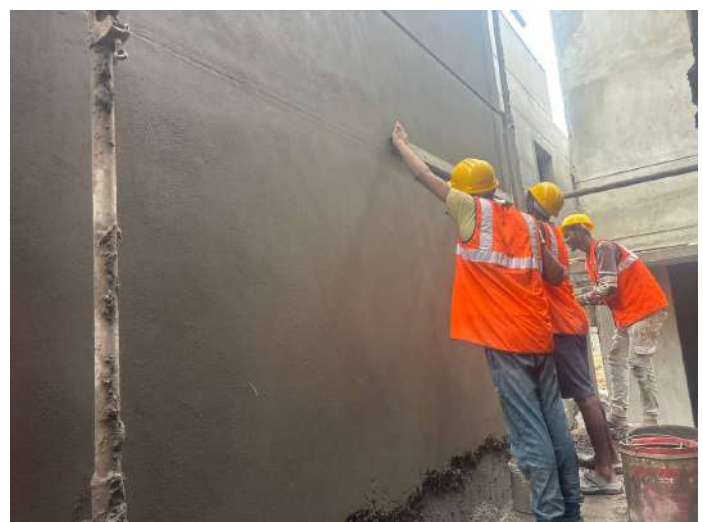
V66 - External Plastering
