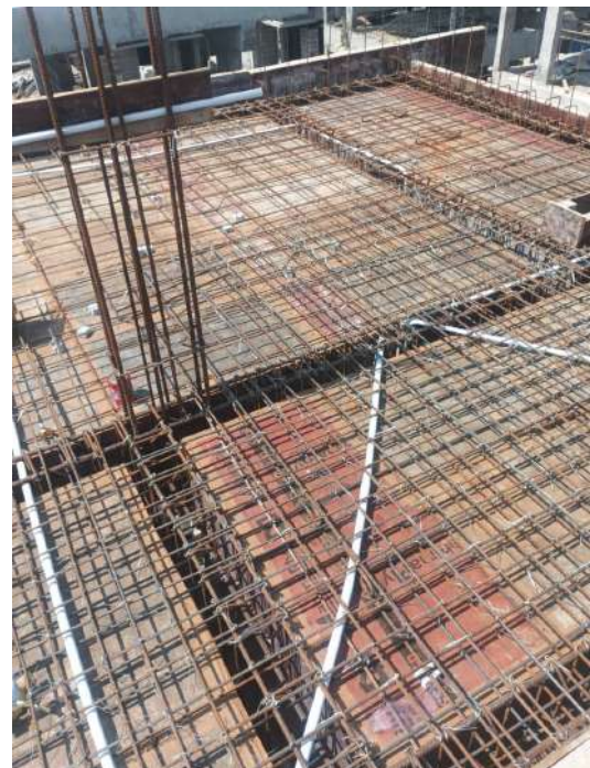
V113 - SF- Roof Slab & Beam - Electrical works
