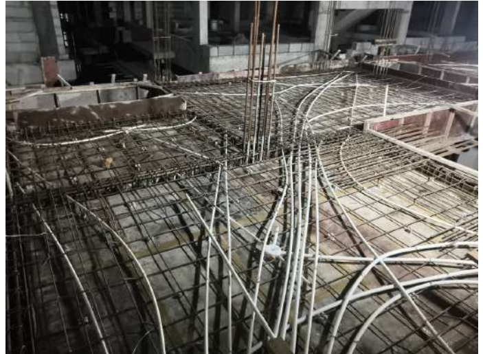
V34 - Ground Floor Roof Slab & Beam - Shuttering, Reinforcement
