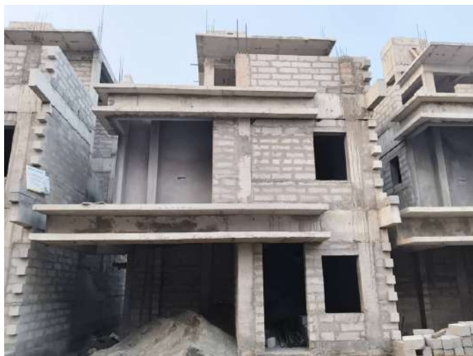
V50 - Internal Plastering
