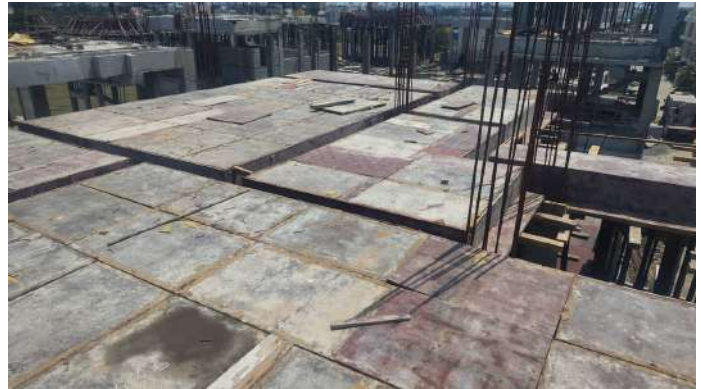
V109 - SF- Roof Slab & Beam - Shuttering, Reinforcement
