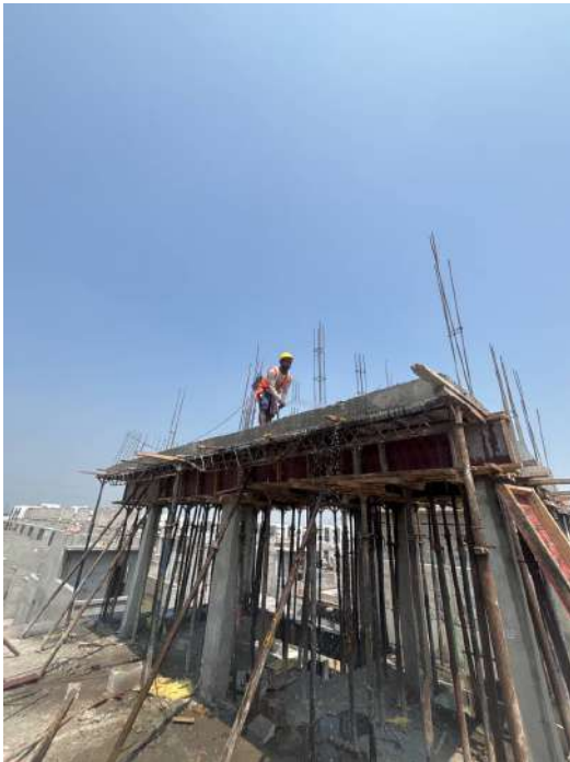
V107 - Stair Head Room Roof Slab & Beam Concreting
