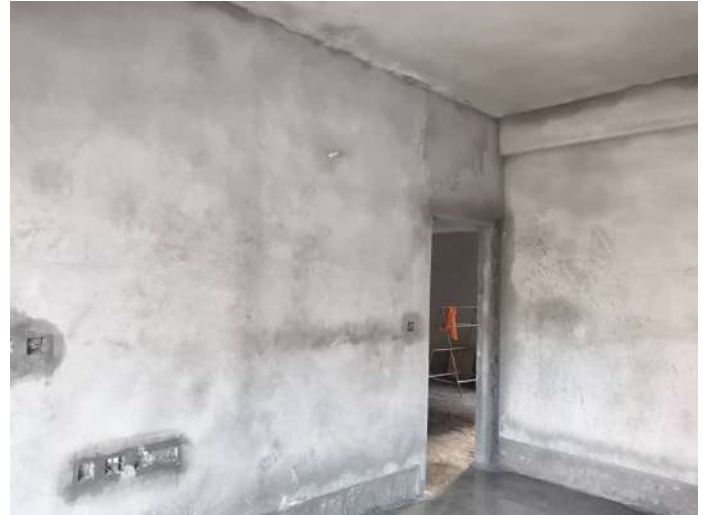
V30 - Internal Plastering
