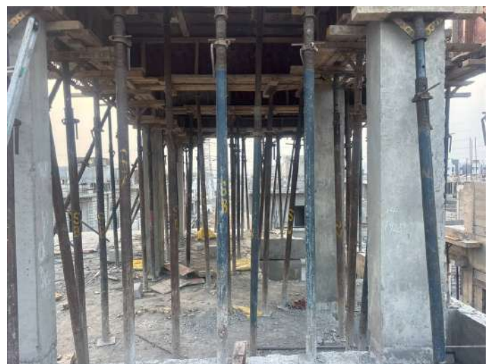
V107 - Stair Head Room Column Concreting
