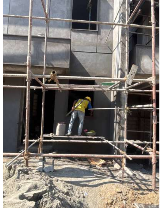
V69 - External Plastering
