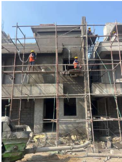
V63 - External Plastering
