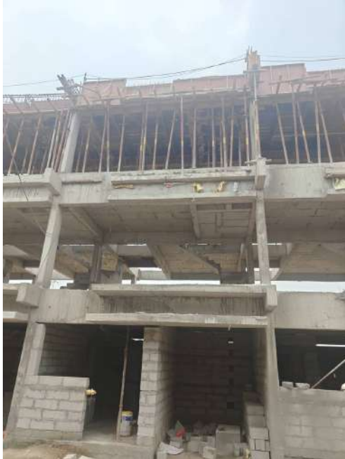
V94 - Completion of Staircase Headroom with Part Roof slab
