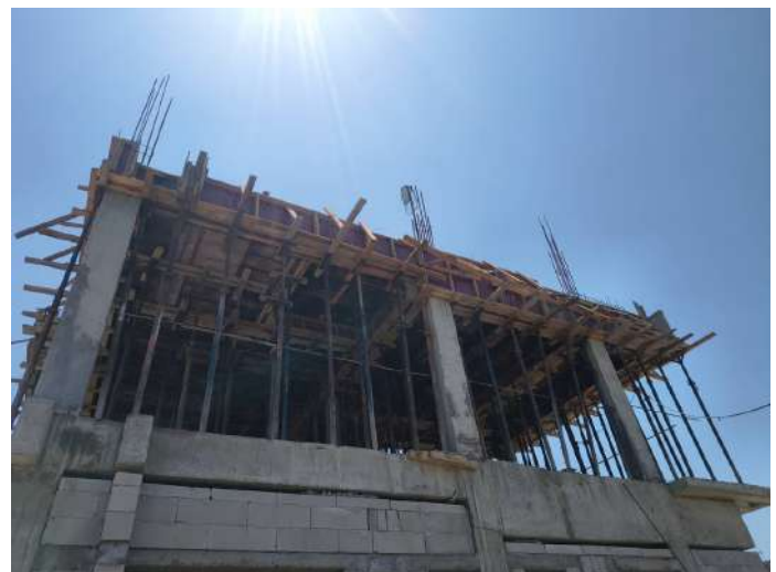
V62 - First Floor Roof Slab & Beam - Shuttering, Reinforcement
