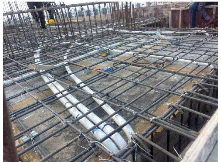
V107 - Stair Head Room Roof Slab & Beam - Electrical works
