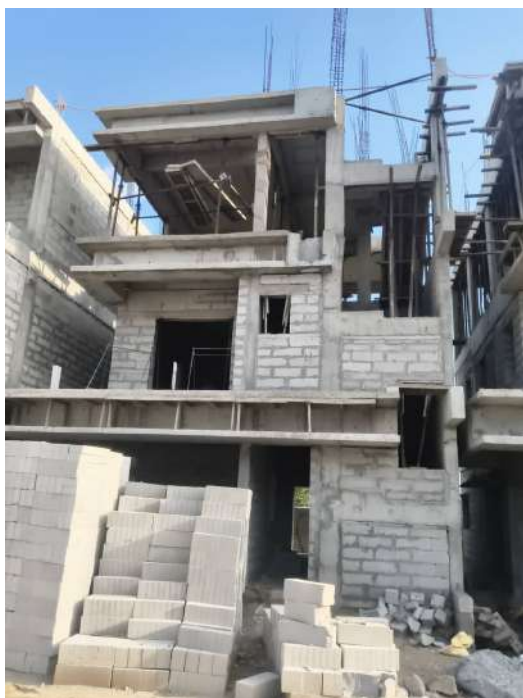
V24 - Completion of Second Floor Roof Slab
