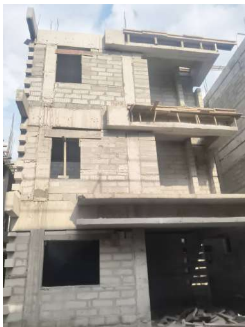
V36 - Completion of Blockwork
