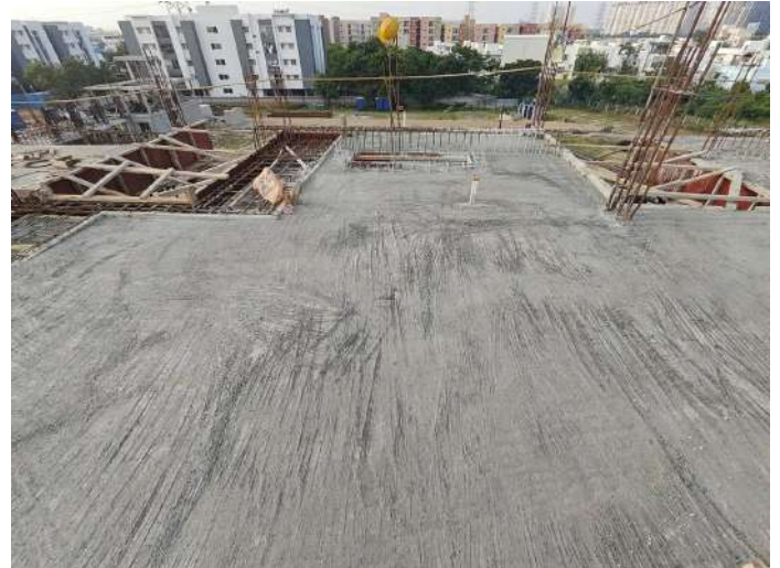
V94 - Stair Headroom with Part Roof Slab & Beam Concreting
