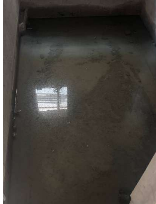
V68 - Toilet Waterproofing
