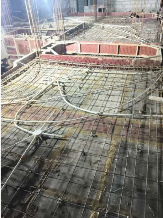
V35 - Ground Floor Roof Slab & Beam - Shuttering, Reinforcement
