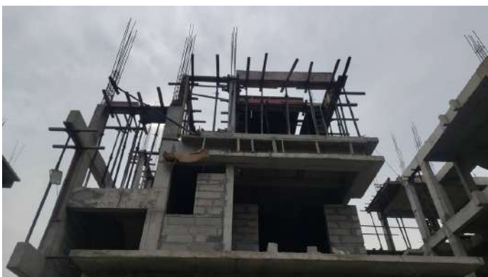
V109 - SF- Roof Slab & Beam - Shuttering, Reinforcement
