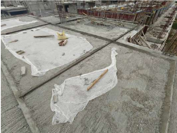
V98 - Completion of Staircase Headroom with Part roof slab
