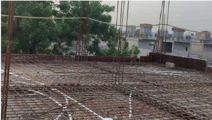
V109 - SF- Roof Slab & Beam - Shuttering, Reinforcement
