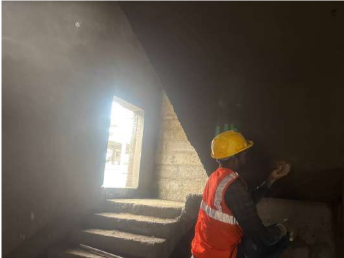
V106 - Internal Plastering
