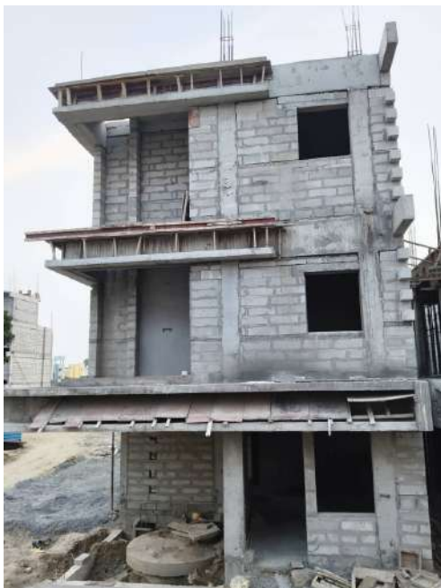
V33 - Instllation of Wall chasing & Electrical conduits
