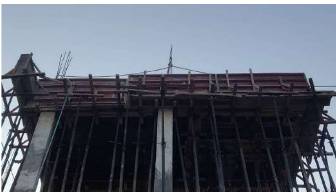
V119 - Staircase Headroom with Part Roof Slab & Beam - Shuttering, Reinforcement
