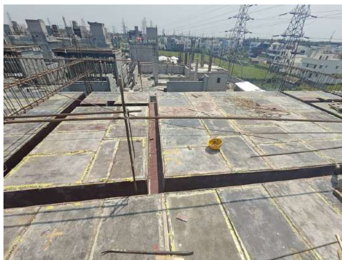
V85 - Stair Head Room Roof Slab & Beam - Shuttering, Reinforcement
