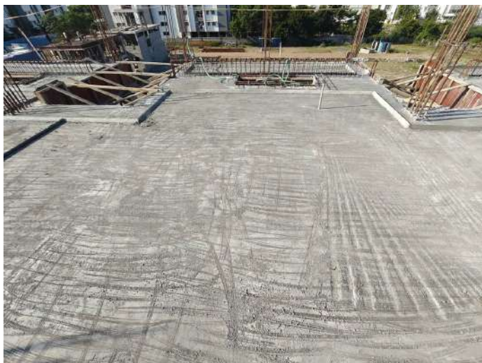
V92 - Stair Head Room Roof Slab & Beam Concreting
