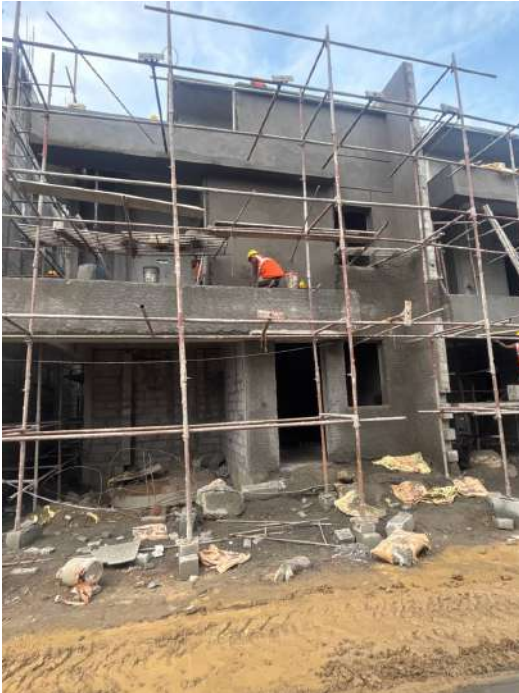
V65 - External Plastering
