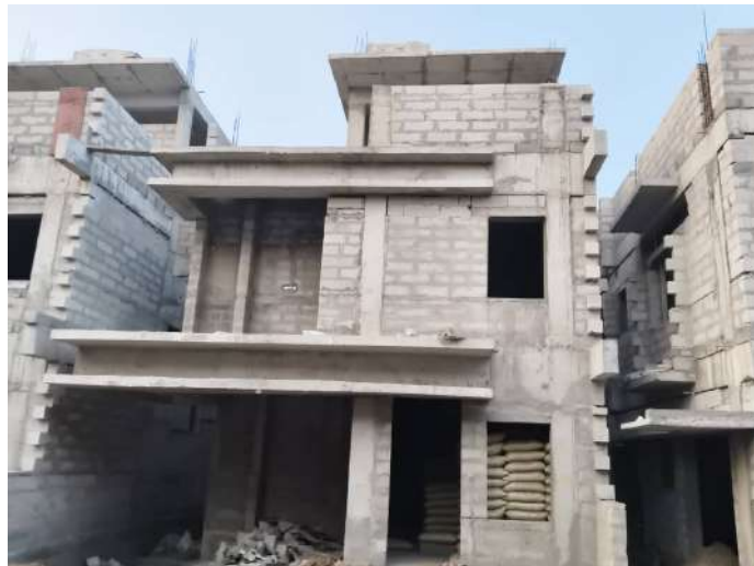
V52 - Internal Plastering
