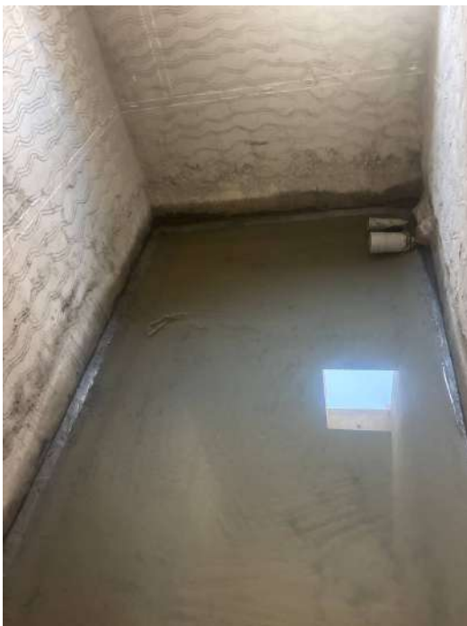
V71 - Toilet Waterproofing
