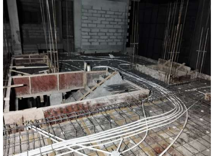
V35 - First Floor Roof Slab & Beam - Shuttering, Reinforcement
