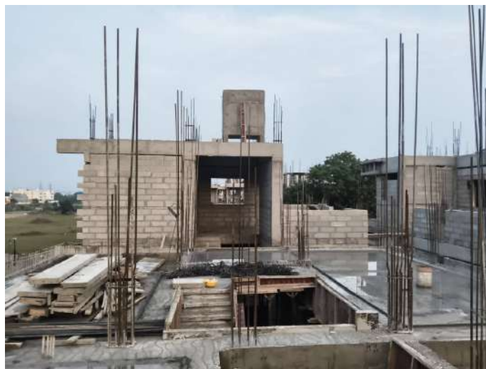
V34 - Completion of First Floor Roof Slab
