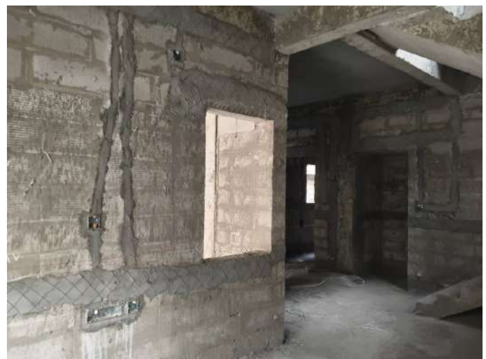
V55 - Instllation of Wall chasing & Electrical conduits
