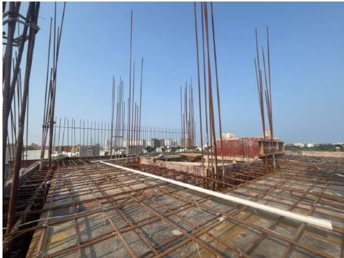
V104 - Stair Head Room Roof Slab & Beam - Shuttering, Reinforcement
