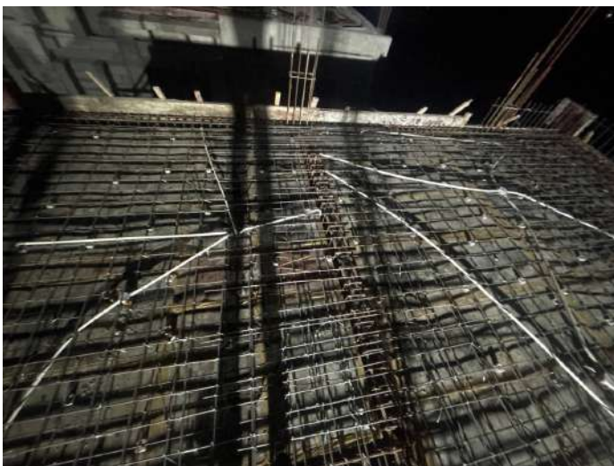
V103 - SF- Roof Slab & Beam - Electrical works
