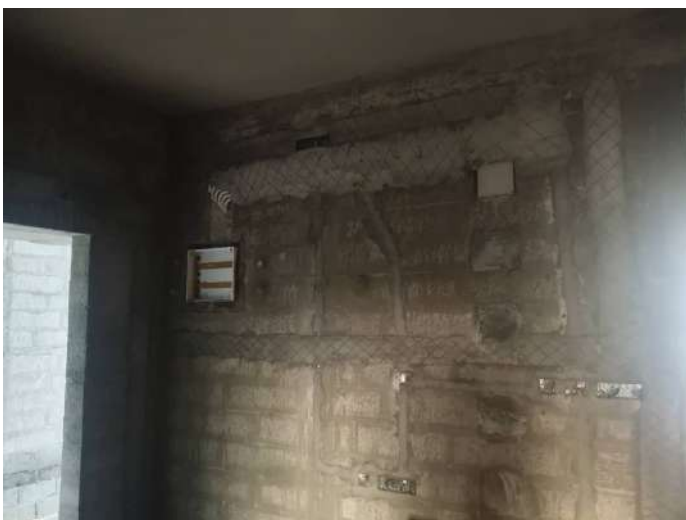
V30 - Instllation of Wall chasing & Electrical conduits
