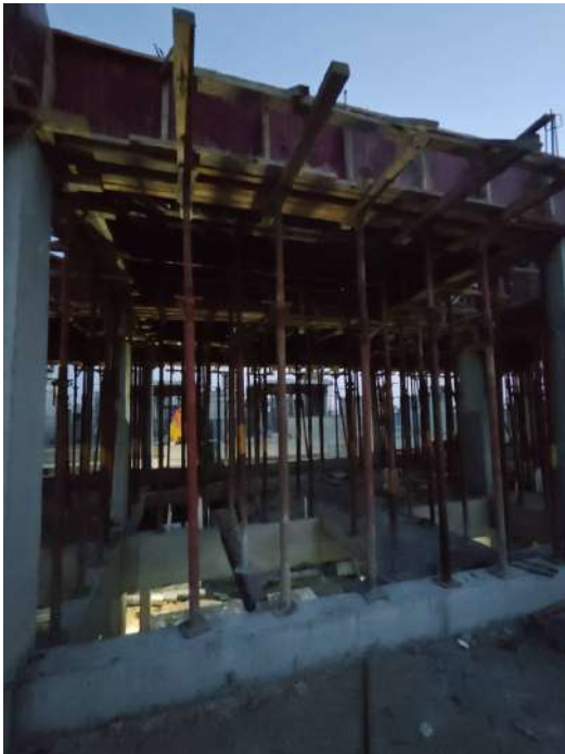
V90 - Stair Head Room Roof Slab & Beam - Shuttering, Reinforcement
