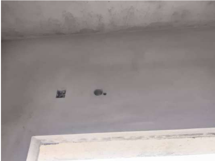
V29 - Internal Plumbing Core Cutting & Wall chasing
