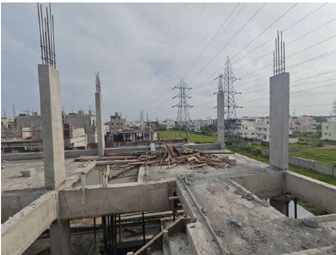
V83 - Stair Head Room Column Concreting
