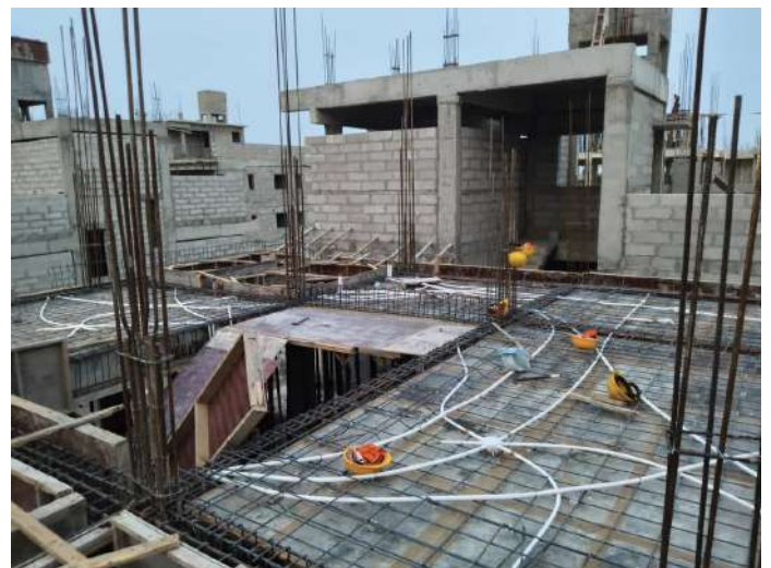
V34 - First Floor Roof Slab & Beam - Electrical works
