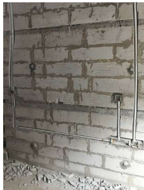
V97 - Instllation of Wall chasing & Electrical conduits
