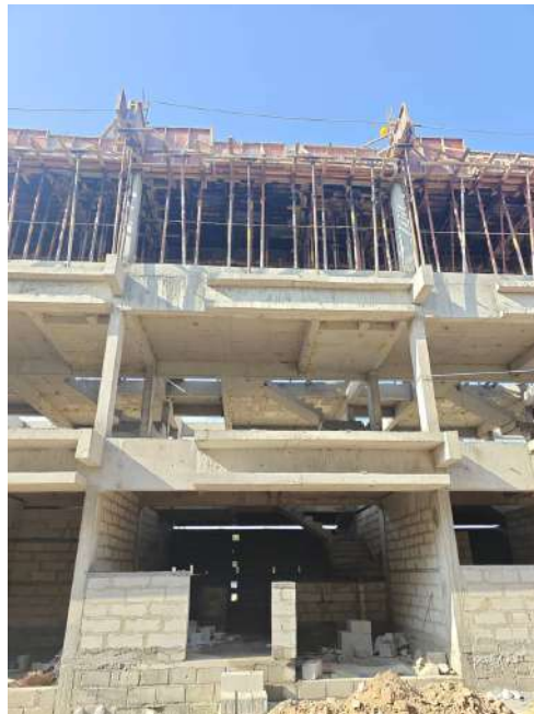
V92 - Stair Head Room Roof Slab & Beam Concreting
