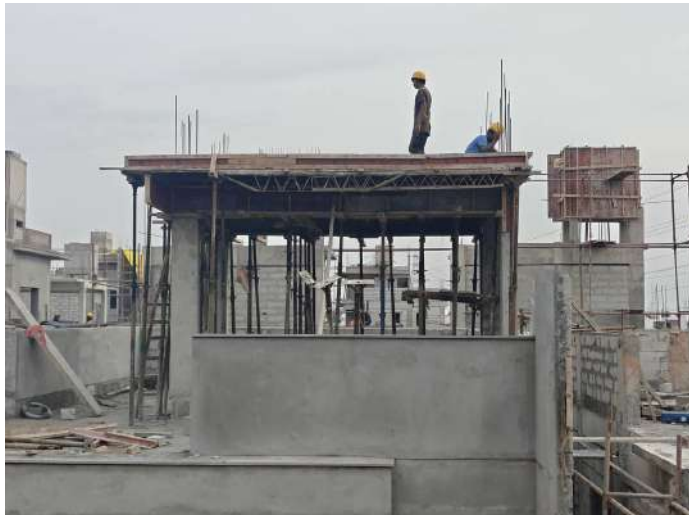
V80 - Stair Head Room Roof Slab & Beam - Shuttering, Reinforcement
