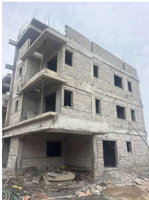
V108 - Completion of Blockwork
