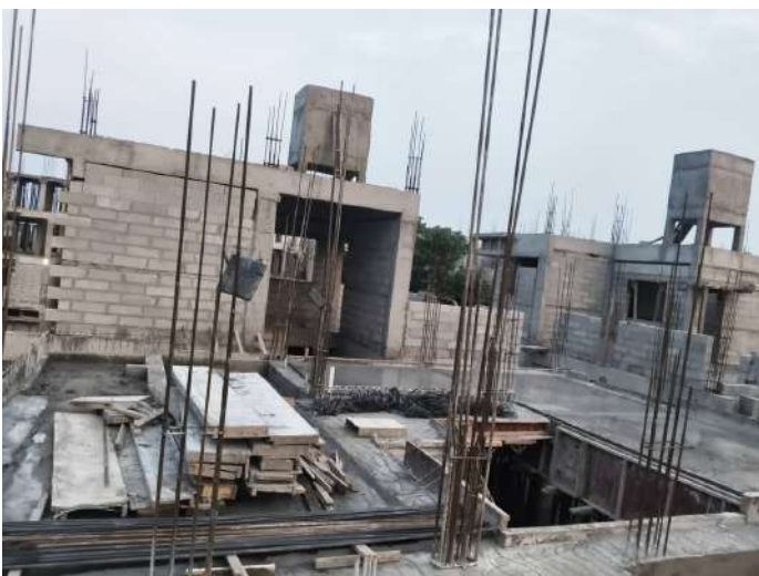
V34 - First Floor Roof Slab & Beam Concreting
