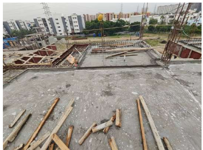
V94 - Completion of Staircase Headroom with Part Roof slab
