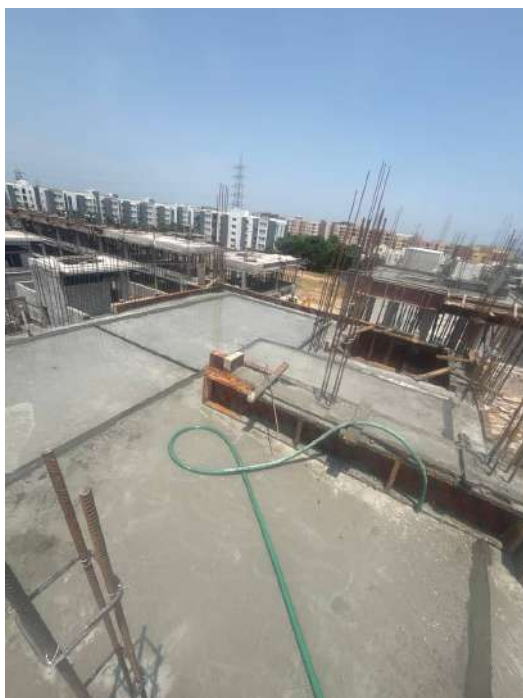
V106 - Stair Head Room Roof Slab & Beam Concreting
