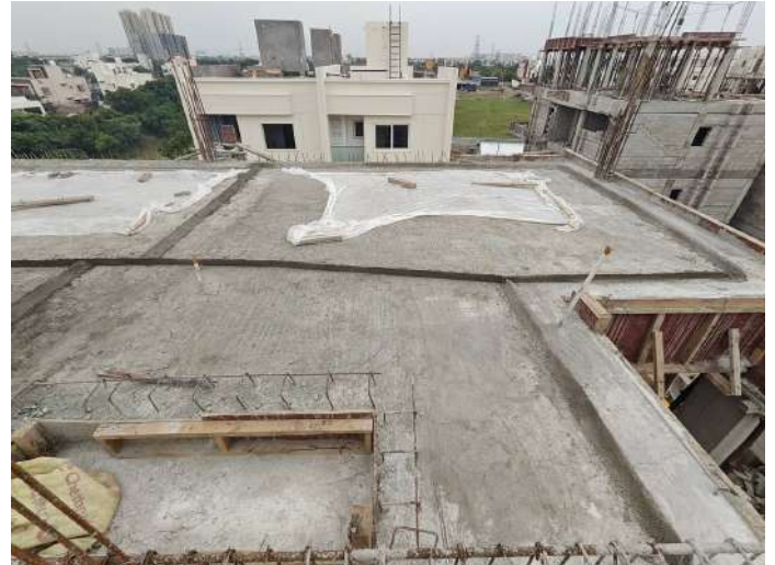
V97 - Completion of Staircase Headroom with Part roof slab
