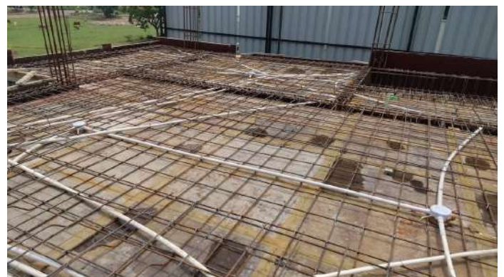
V123 - Ground Floor Roof Slab & Beam - Shuttering, Reinforcement
