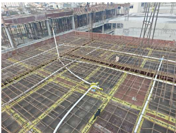
V78 - Stair Head Room Roof Slab & Beam - Shuttering, Reinforcement
