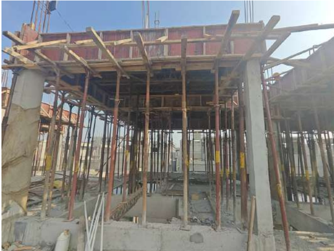
V96 - Staircase Headroom with Part Roof Slab & Beam - Shuttering, Reinforcement
