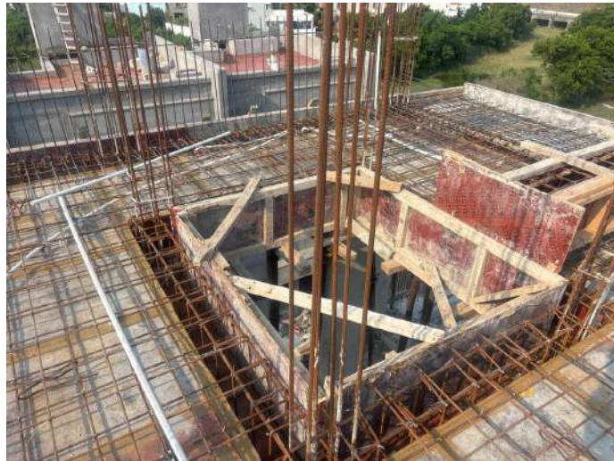
V104 - Stair Head Room Roof Slab & Beam - Electrical works
