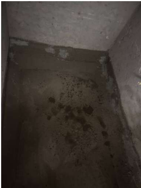
V70 - Toilet Waterproofing
