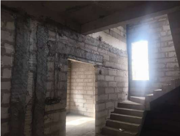
V36 - Completion of Blockwork
