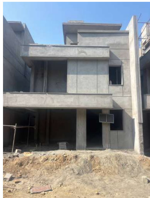
V69 - External Plastering
