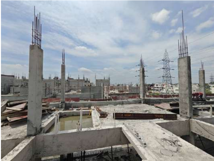
V86 - Stair Head Room Column Concreting
