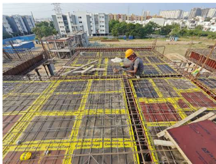
V90 - Stair Head Room Roof Slab & Beam - Shuttering, Reinforcement
