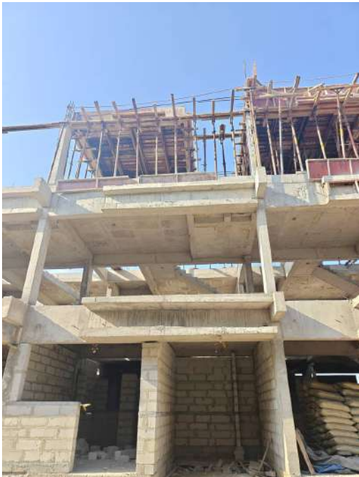
V88 - Stair Head Room Roof Slab & Beam - Shuttering, Reinforcement
