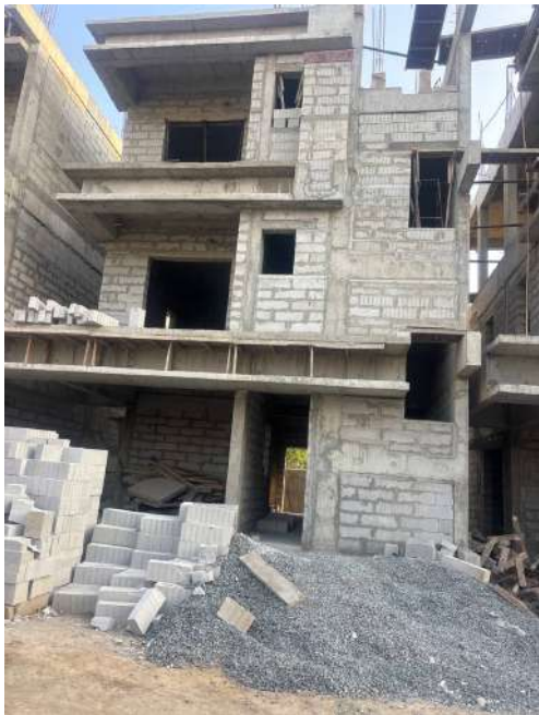
V23 - Completion of Blockwork
