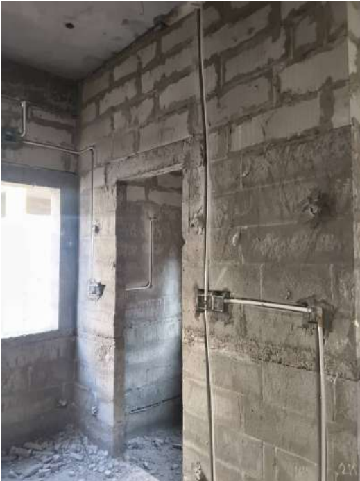
V56 - Instllation of Wall chasing & Electrical conduits
