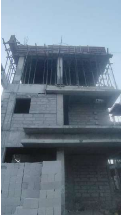
V119 - Stair Head Room with Part Roof Slab & Beam Concreting
