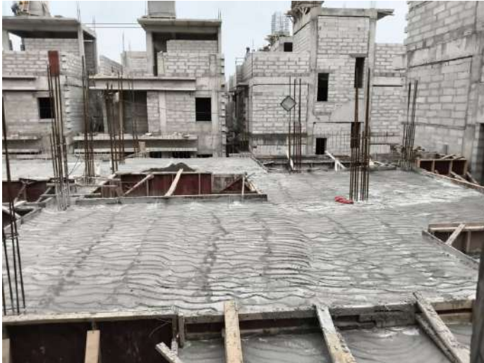
V34 - Completion of Ground Floor Roof Slab
