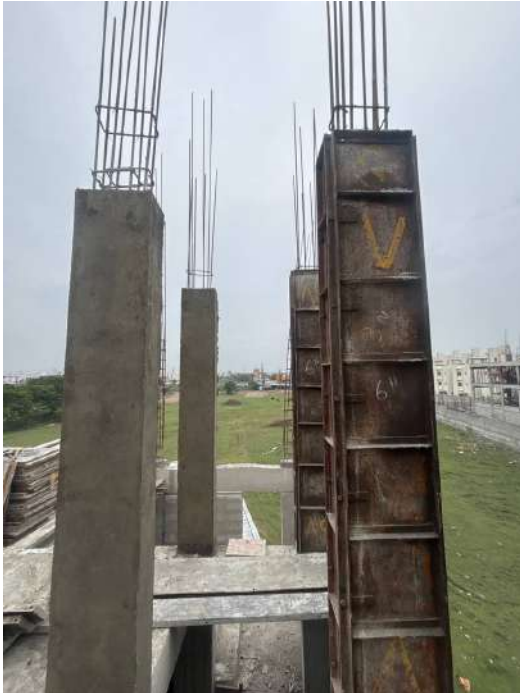
V103 - SF- Column Concreting
