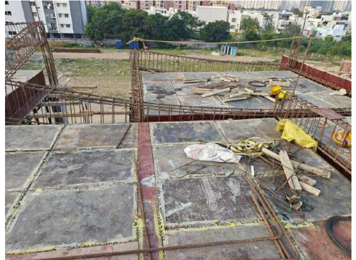
V93 - Stair Head Room Roof Slab & Beam - Shuttering, Reinforcement
