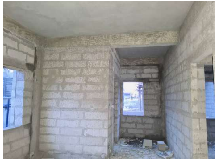
V30 - Completion of Blockwork
