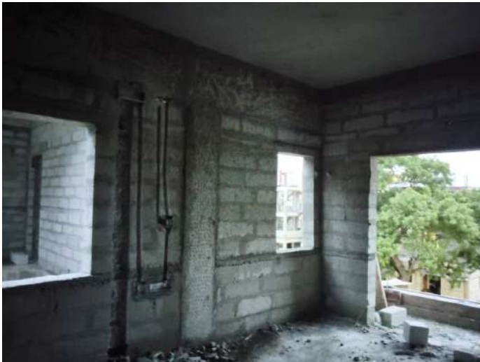
V30 - Completion of Blockwork
