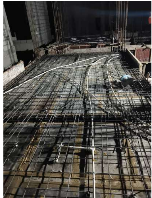
V34 - First Floor Roof Slab & Beam - Shuttering, Reinforcement
