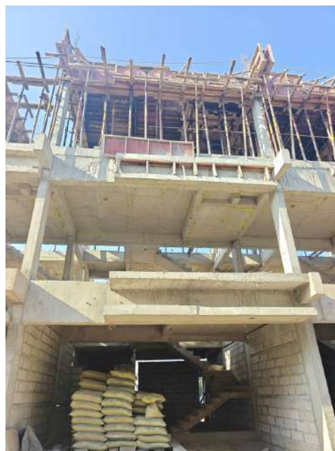
V89 - Completion of Staircase Headroom & Part Roof Slab
