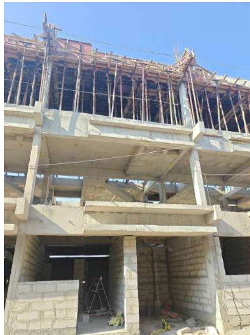
V93 - Completion of Staircase Headroom & Part Roof Slab
