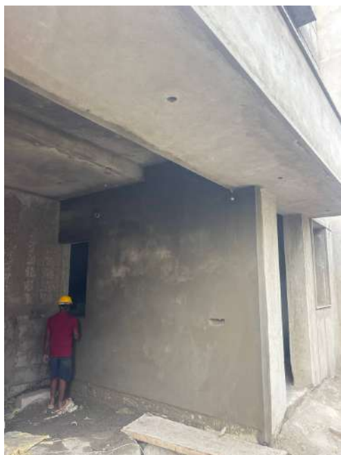
V66 - External Plastering
