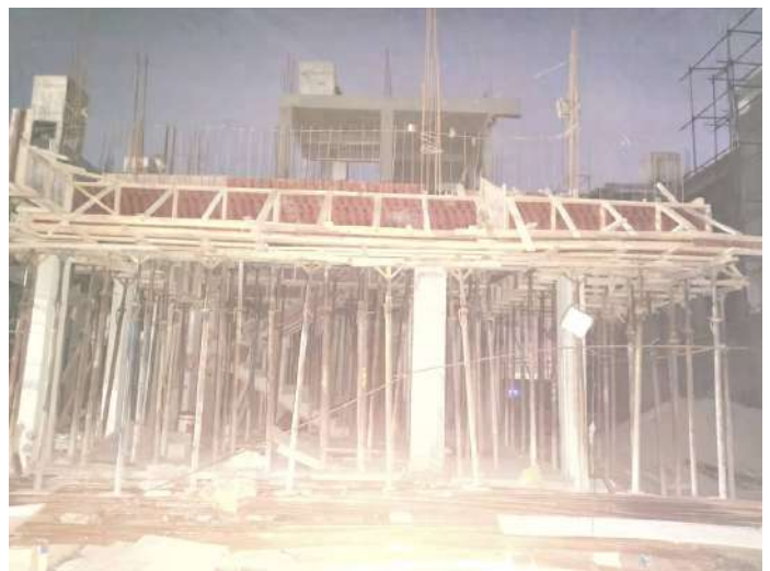
V35 - Ground Floor Roof Slab & Beam - Shuttering, Reinforcement
