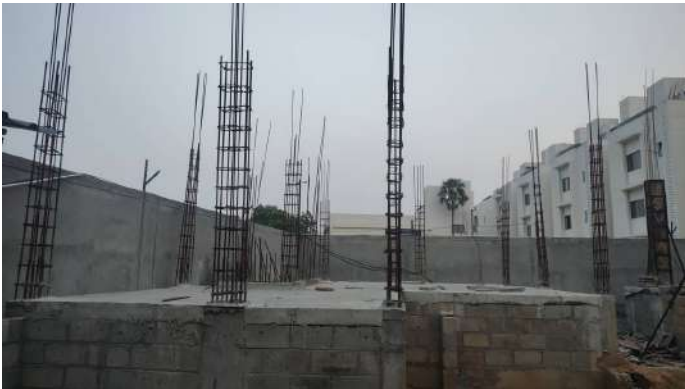
V121 - UG Sump - Excavation & Erection
