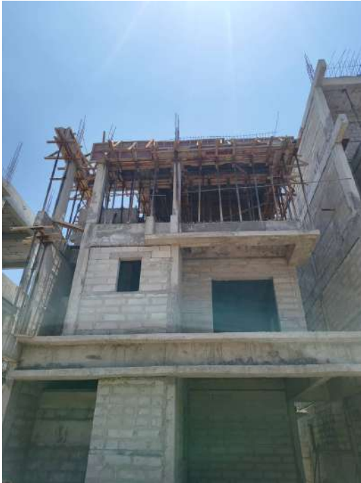
V107 - SF- Roof Slab & Beam Concreting
