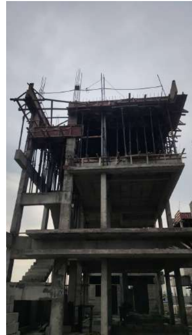
V113 - SF- Roof Slab & Beam Concreting
