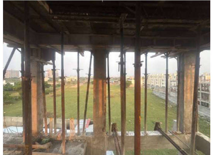
V103 - Stair Head Room Column Concreting
