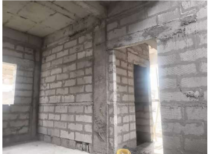
V36 - Completion of Blockwork
