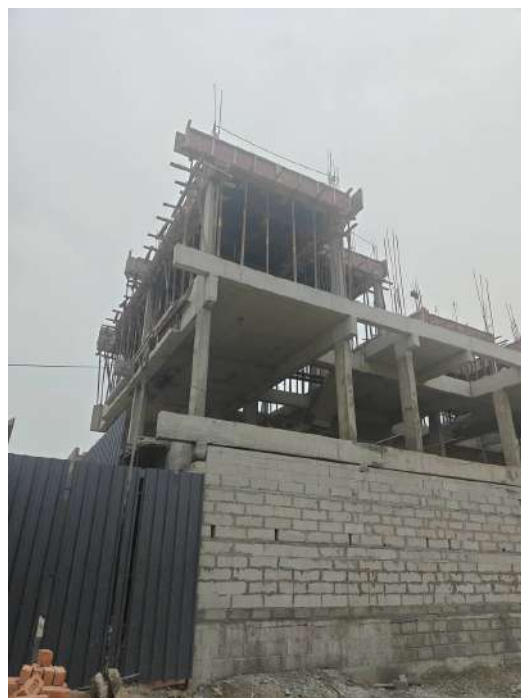
V98 - Completion of Staircase Headroom with Part roof slab
