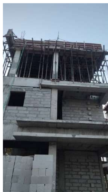
V119 - Completion of Staircase Headroom with Part roof slab
