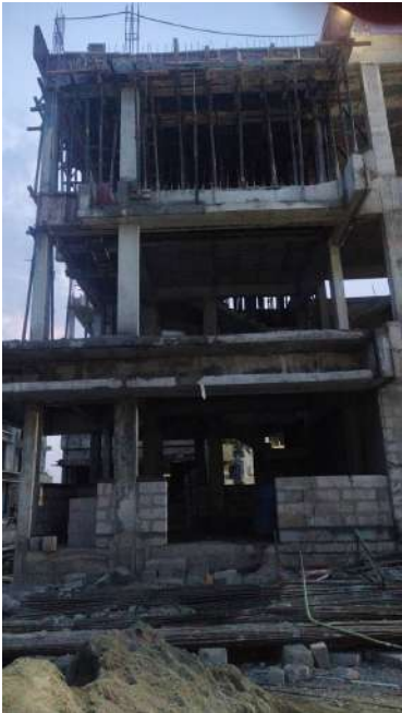
V117 - Completion of Second Floor Roof Slab
