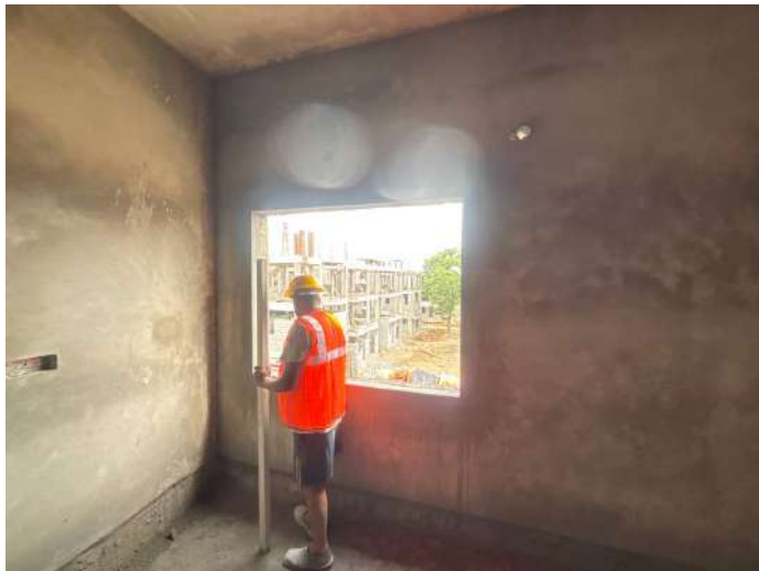
V108 - Internal Plastering
