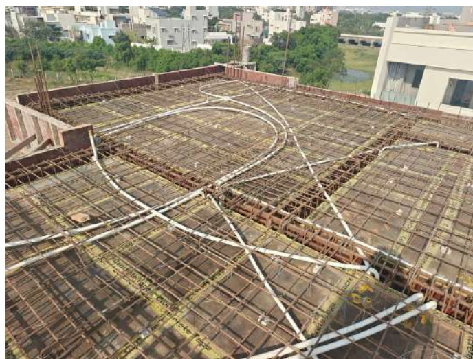
V98 - Staircase Headroom Roof Slab & Beam - Shuttering, Reinforcement
