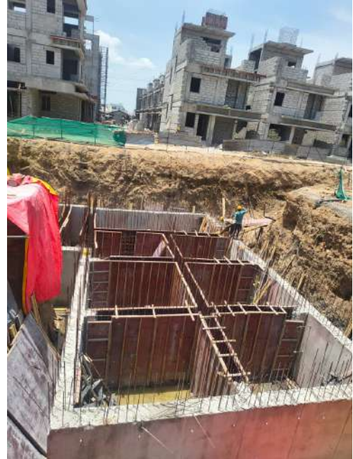
STP - Civil works
