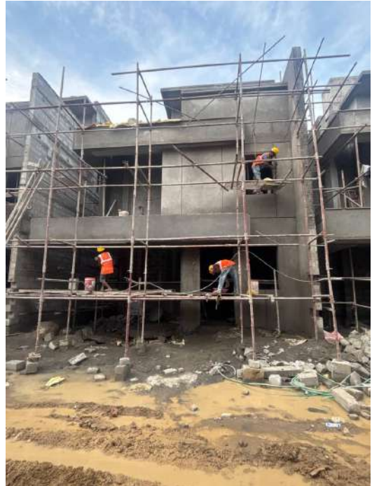
V66 - External Plastering
