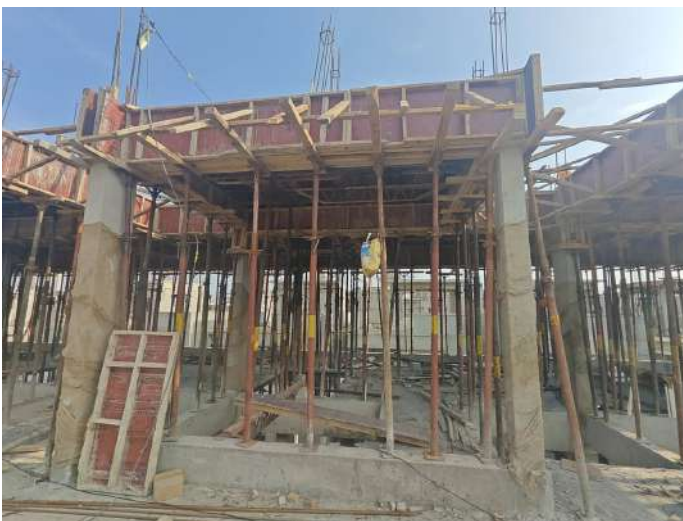
V94 - Stair Headroom with Part Roof Slab & Beam - Shuttering, Reinforcement
