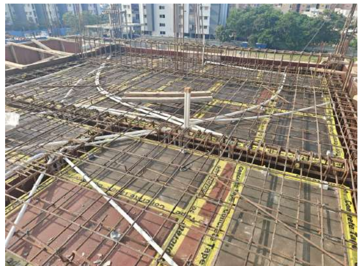
V94 - Stair Headroom with Part Roof Slab & Beam - Electrical works
