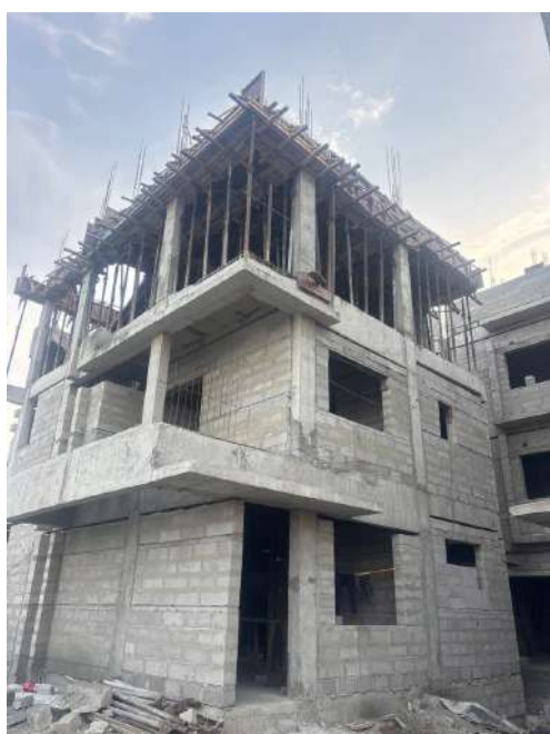
V103 - Completion of Second Floor Roof Slab
