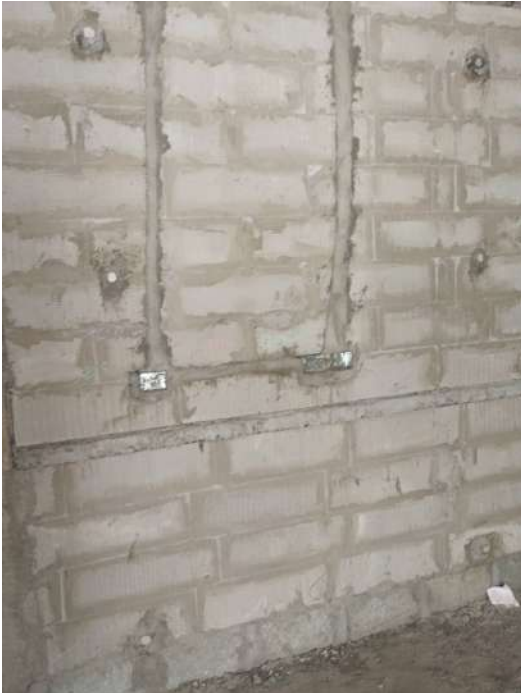
V104 - Instillation of Wall chasing & Electrical conduits
