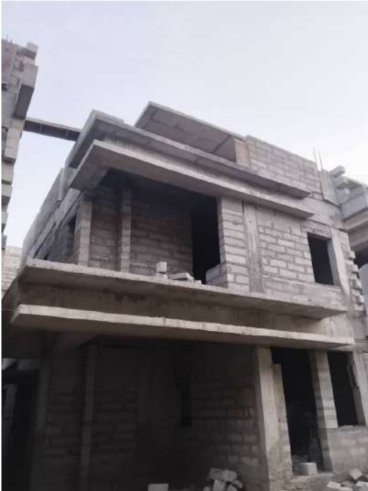
V58 - Completion of Blockwork
