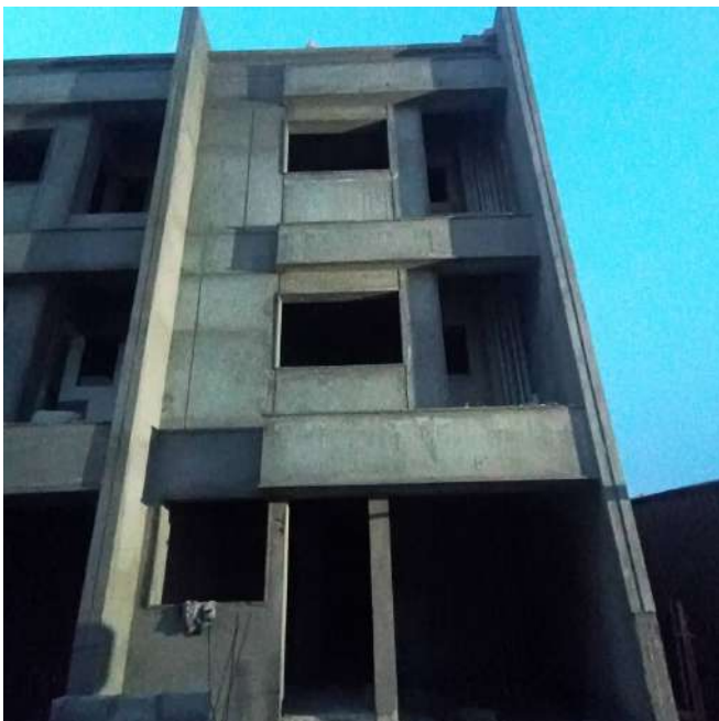
V102 - External Plastering
