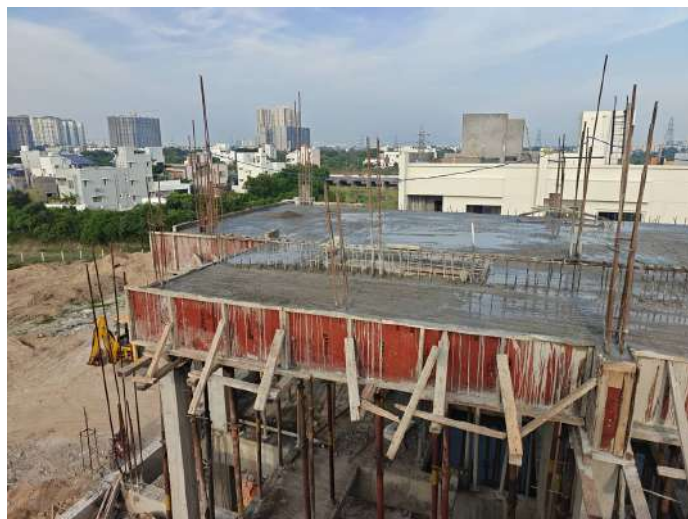
V98 - Staircase Headroom with Part Roof Slab & Beam Concreting
