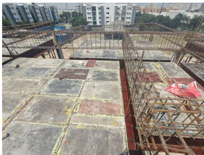
V87 - Stair Head Room Roof Slab & Beam - Shuttering, Reinforcement
