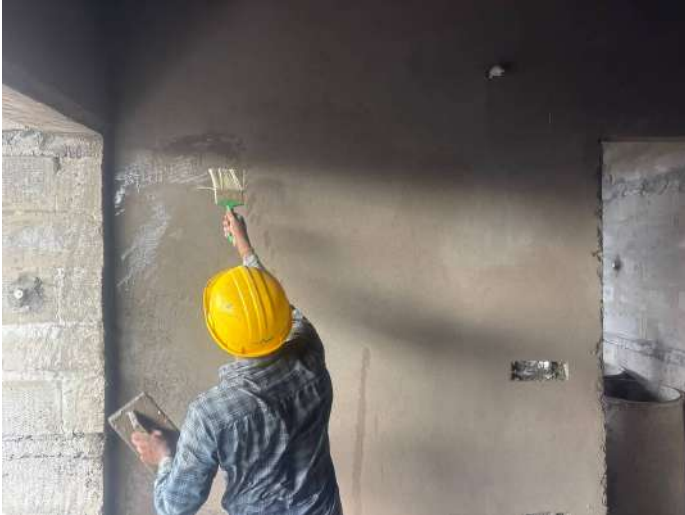
V106 - Internal Plastering
