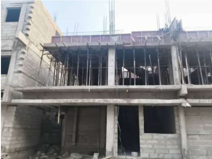
V34 - First Floor Roof Slab & Beam Concreting
