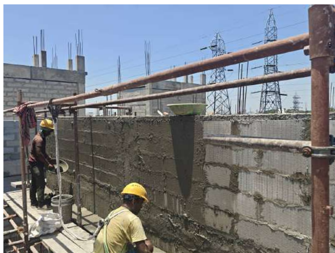
V80 - External Plastering
