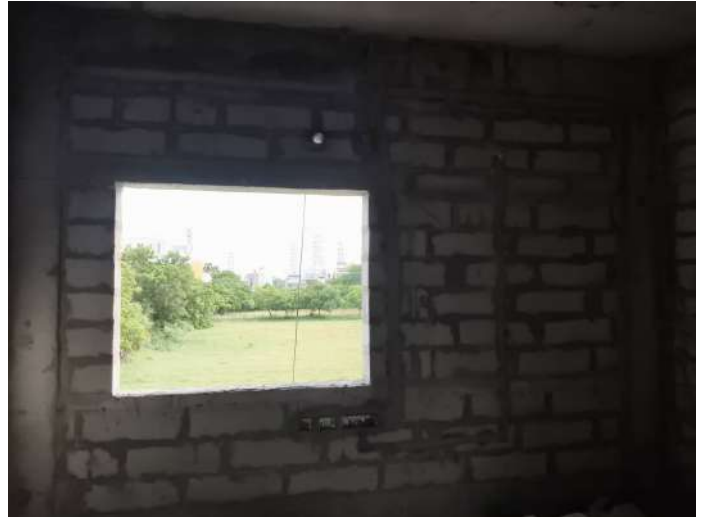
V23 - Completion of Blockwork
