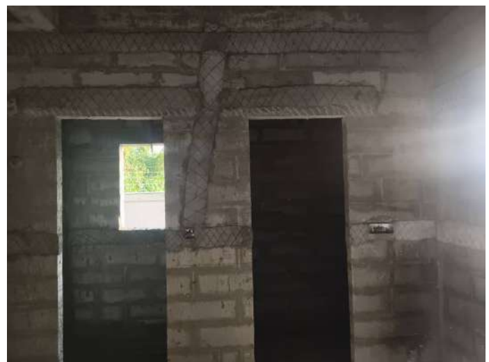
V30 - Instllation of Wall chasing & Electrical conduits
