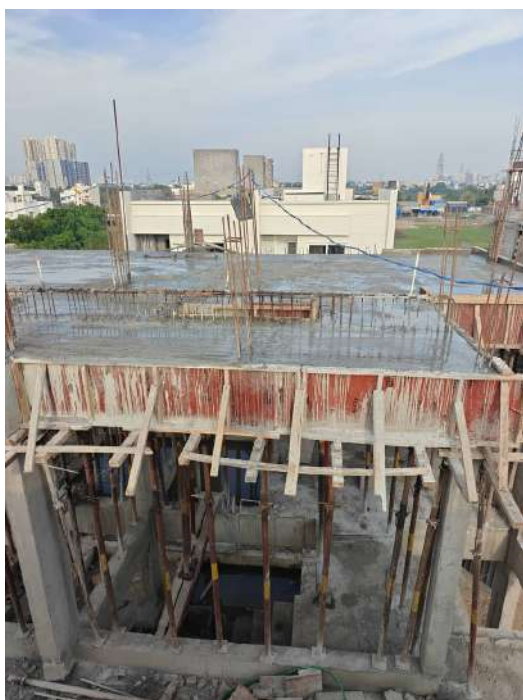
V97 - Staircase Headroom with Part Roof Slab & Beam Concreting
