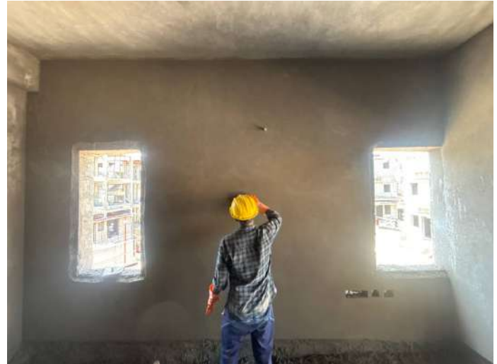
V108 - Internal Plastering
