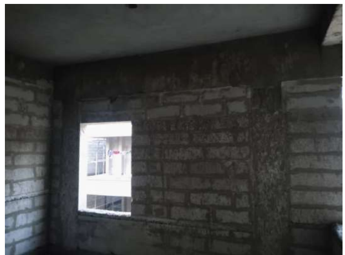
V58 - Completion of Blockwork
