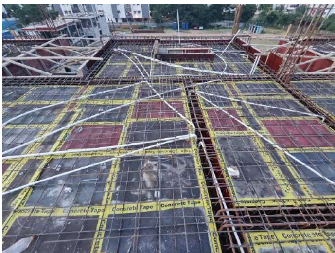
V91 - Stair Head Room Roof Slab & Beam - Electrical works
