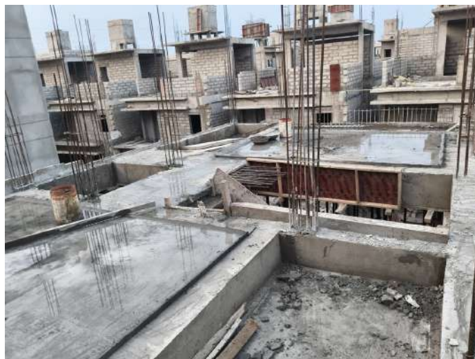
V35 - Completion of First Floor Roof Slab
