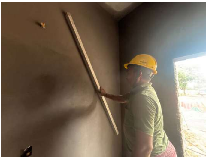
V108 - Internal Plastering
