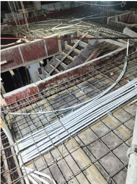
V35 - Ground Floor Roof Slab & Beam - Electrical works
