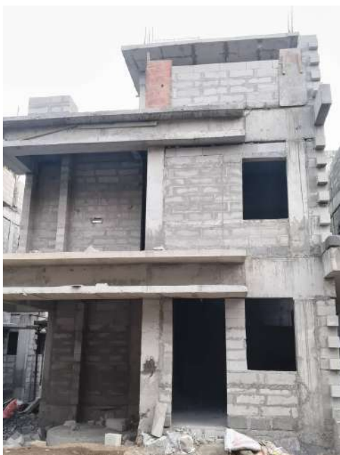
V59 - Completion of Blockwork
