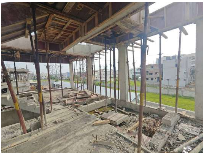
V83 - First Floor Column Concreting
