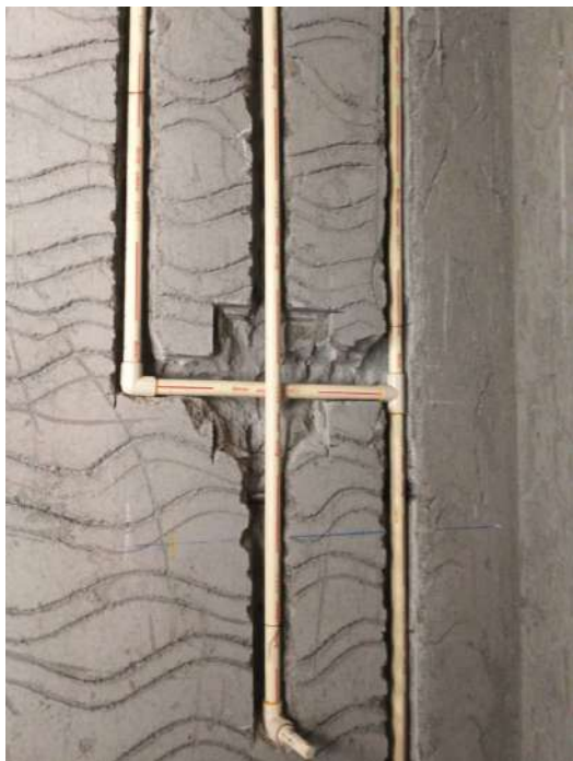
V40 - Internal Plumbing Core Cutting & Wall chasing
