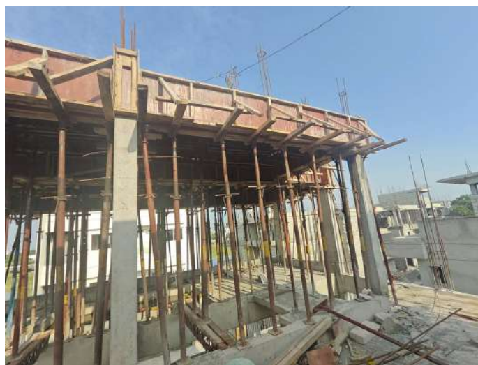
V97 - Staircase Headroom with Part Roof Slab & Beam - Shuttering, Reinforcement
