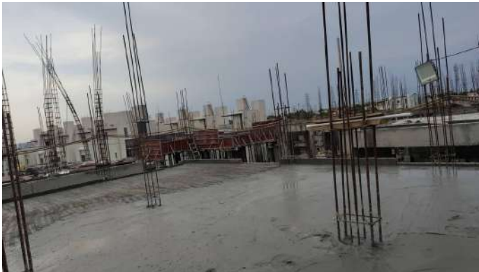
V113 - SF- Roof Slab & Beam Concreting
