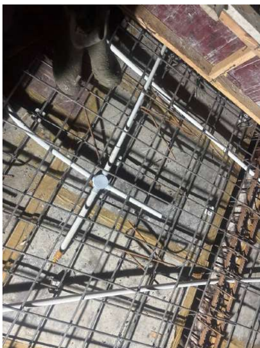
V106 - Stair Head Room Roof Slab & Beam - Electrical works
