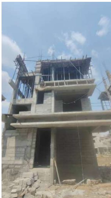
V109 - Completion of Second Floor Roof Slab
