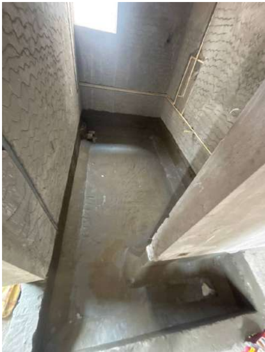
V70 - Toilet Waterproofing
