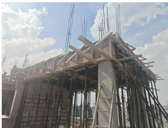
V78 - Stair Head Room Roof Slab & Beam - Shuttering, Reinforcement
