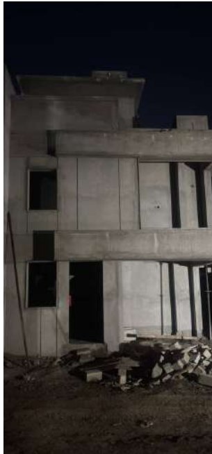
V71 - External Plastering
