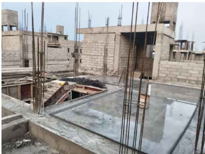
V34 - Completion of First Floor Roof Slab
