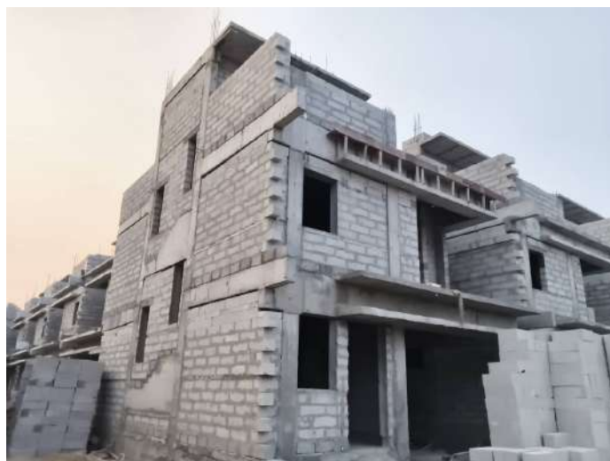
V53 - Instllation of Wall chasing & Electrical conduits
