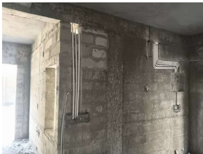
V57 - Completion of Blockwork
