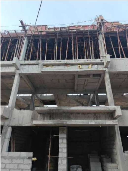
V94 - Stair Headroom with Part Roof Slab & Beam Concreting
