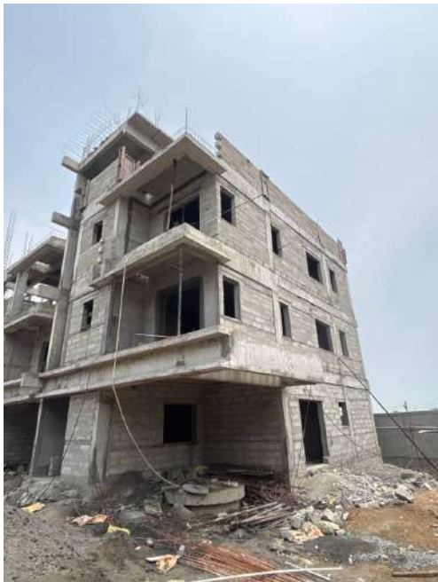
V108 - Completion of Blockwork
