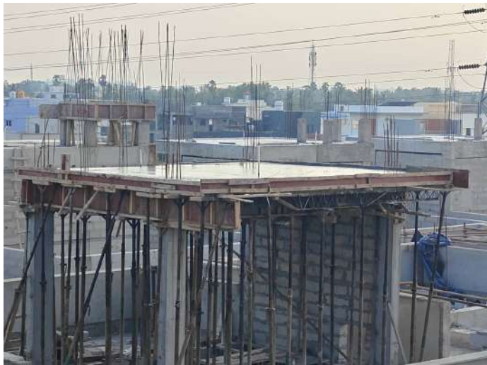
V78 - Stair Head Room Roof Slab & Beam Concreting
