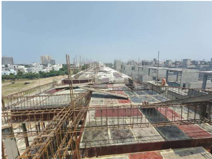
V88 - Stair Head Room Roof Slab & Beam - Shuttering, Reinforcement
