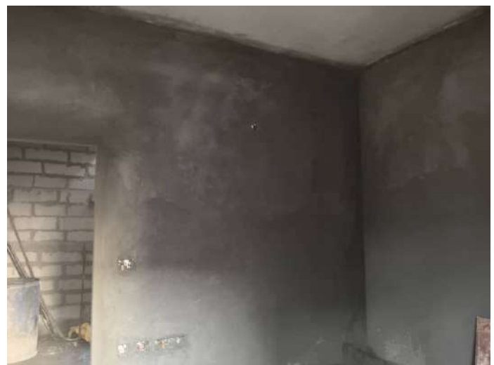
V30 - Internal Plastering
