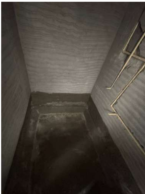
V69 - Toilet Waterproofing
