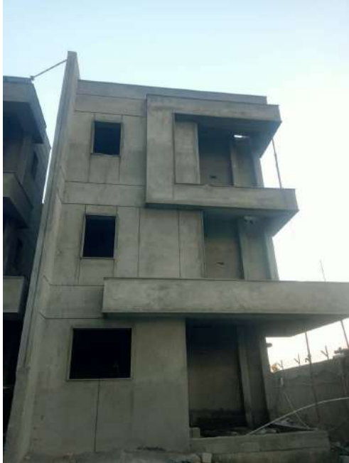
V45 - External Plastering
