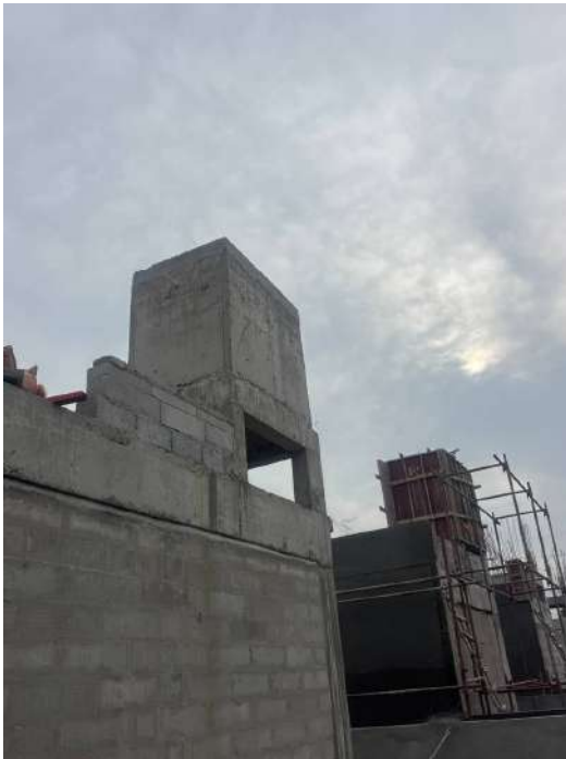
V69 - OHT Waterproofing
