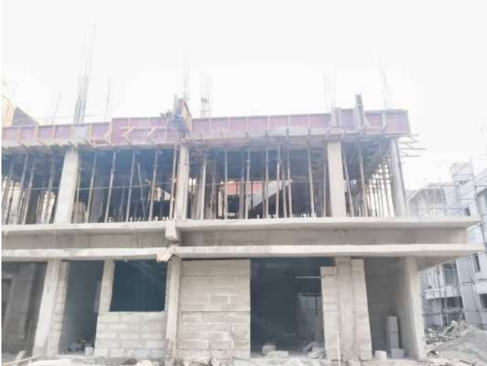
V35 - First Floor Roof Slab & Beam Concreting
