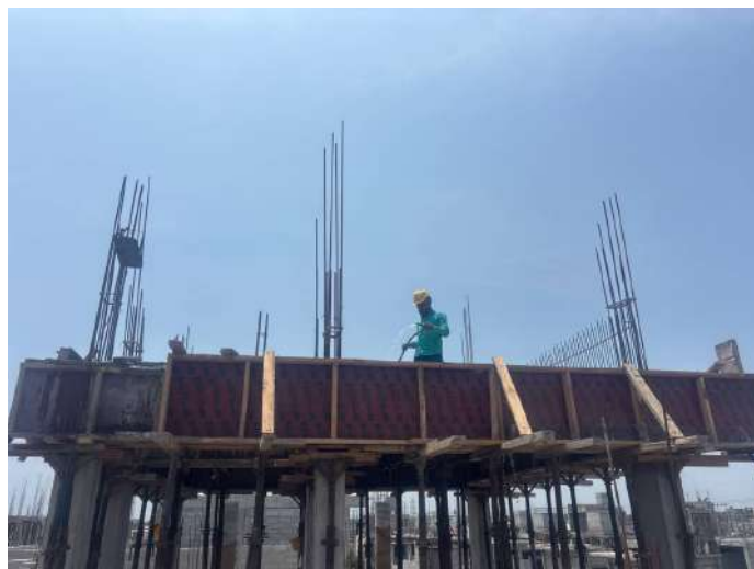
V106 - Stair Head Room Roof Slab & Beam Concreting
