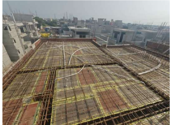
V97 - Staircase Headroom with Part Roof Slab & Beam - Shuttering, Reinforcement
