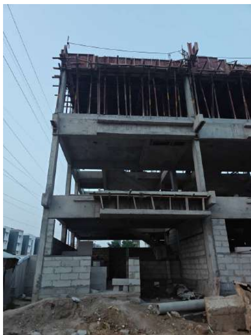
V83 - Stair Head Room Roof Slab & Beam - Shuttering, Reinforcement
