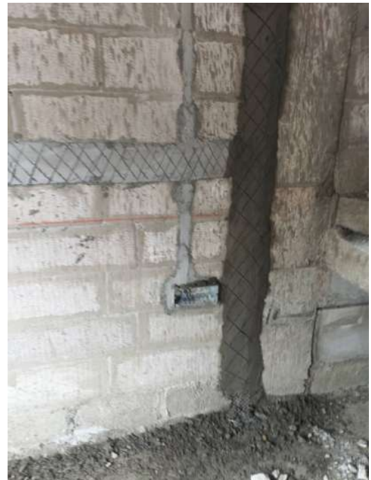
V31 - Instllation of Wall chasing & Electrical conduits
