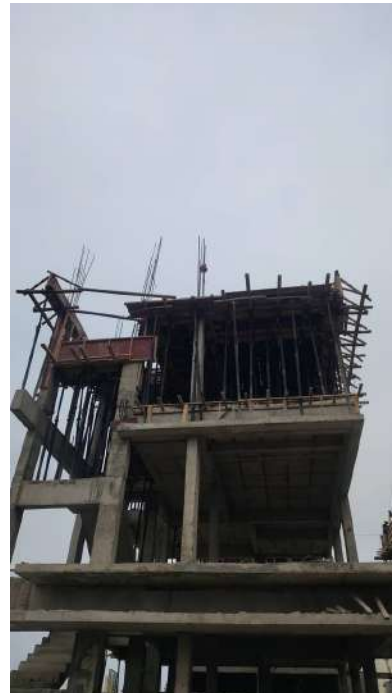
V113 - SF- Roof Slab & Beam - Shuttering, Reinforcement
