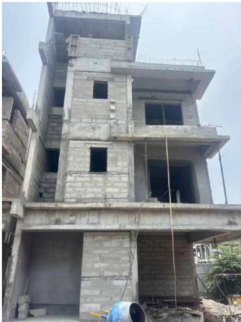
V108 - Completion of Blockwork
