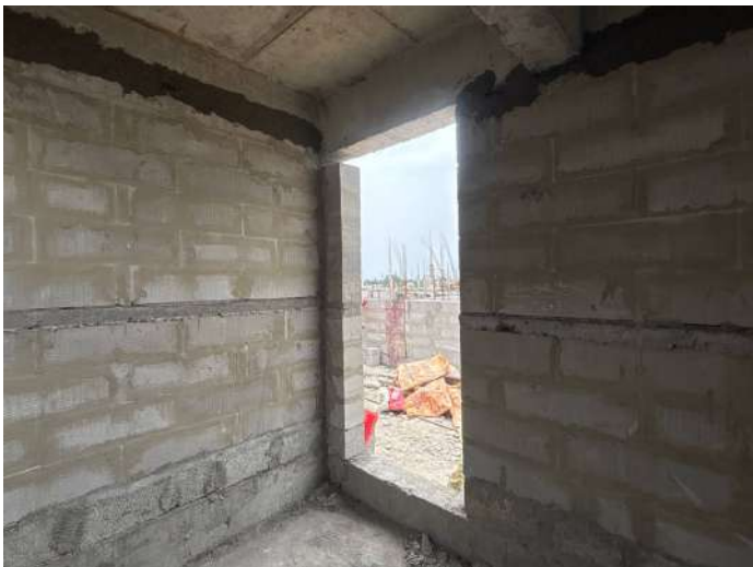
V108 - Completion of Blockwork
