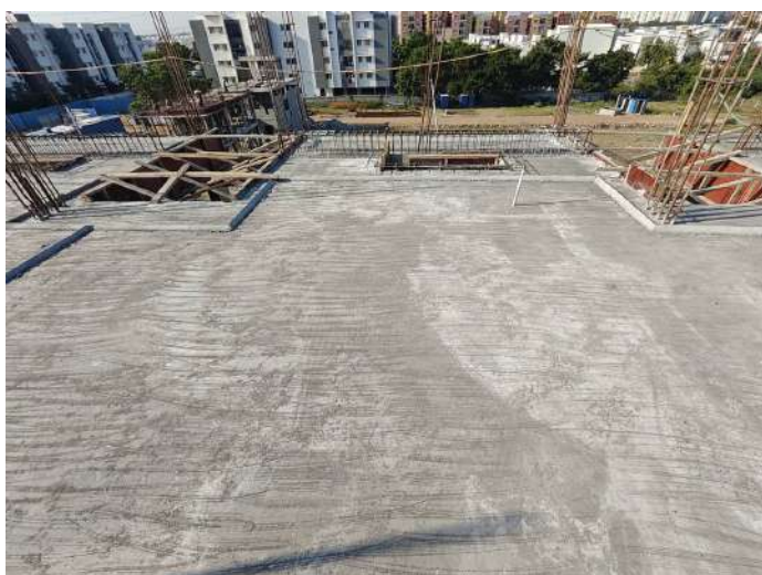
V91 - Completion of Staircase Headroom & Part Roof Slab
