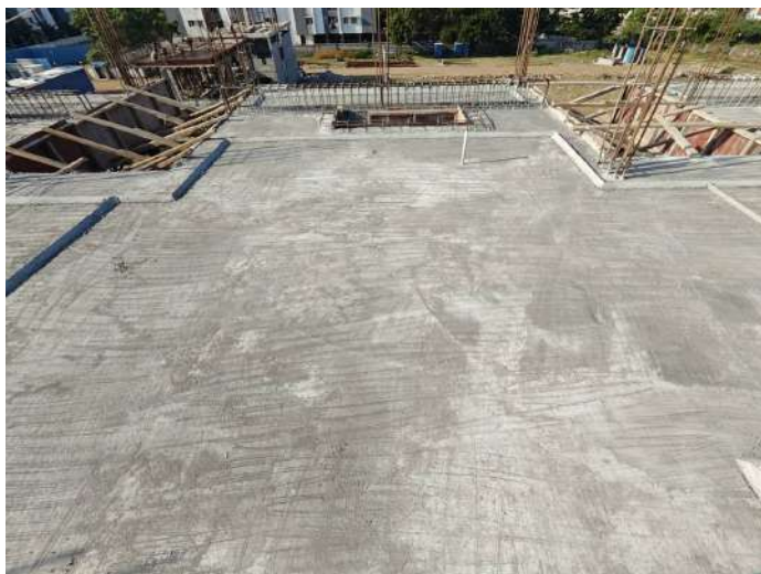
V90- Completion of Staircase Headroom & Part Roof Slab
