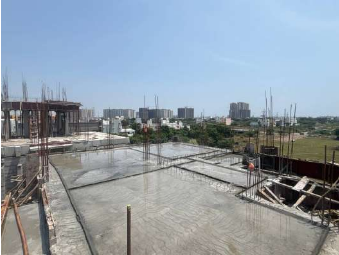
V103 - Completion of Second Floor Roof Slab
