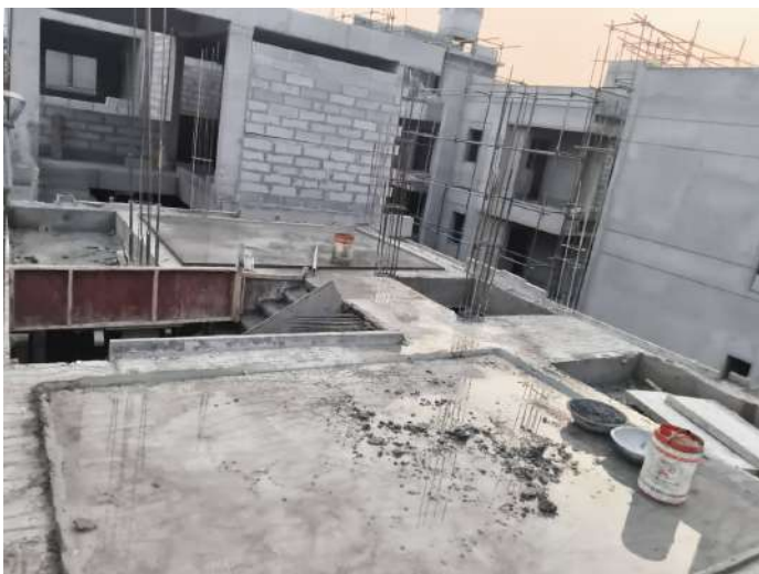
V35 - Completion of First Floor Roof Slab
