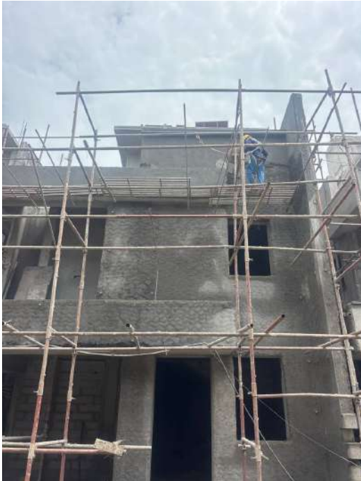
V68 - External Plastering
