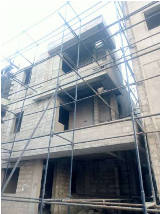
V37 - External Plastering
