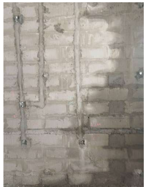
V104 - Instllation of Wall chasing & Electrical conduits
