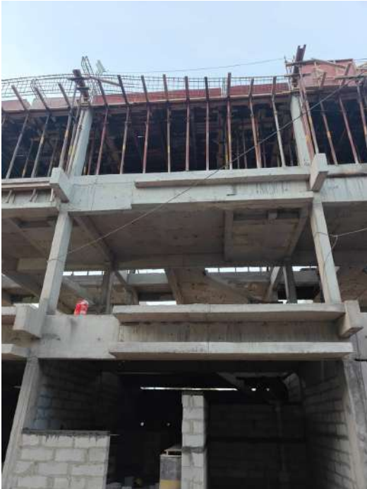
V93 - Stair Head Room Roof Slab & Beam - Shuttering, Reinforcement
