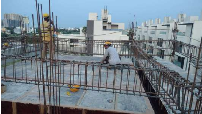
V117 - SF- Roof Slab & Beam - Shuttering, Reinforcement
