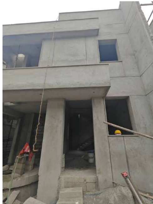
V73 - External Plastering
