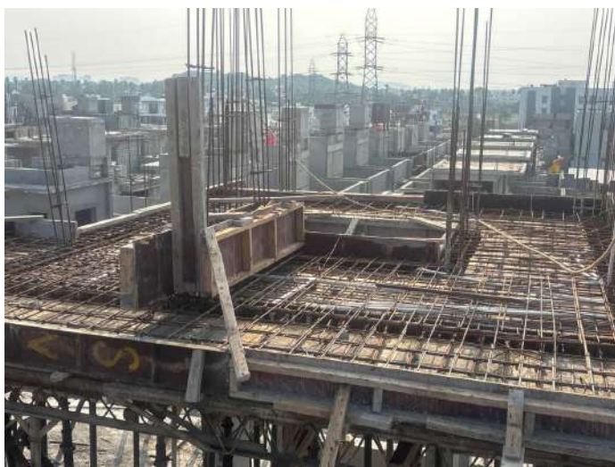
V105 - Stair Head Room Roof Slab & Beam - Electrical works
