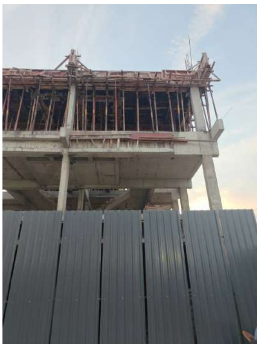
V98 - Staircase Headroom with Part Roof Slab & Beam Concreting
