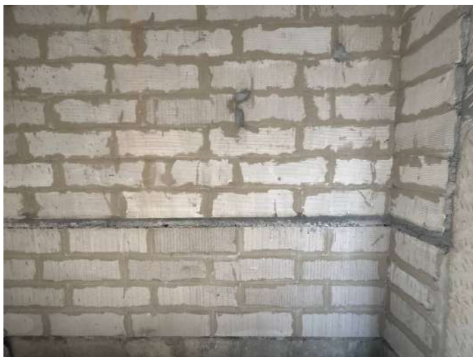
V81 - Completion of Blockwork
