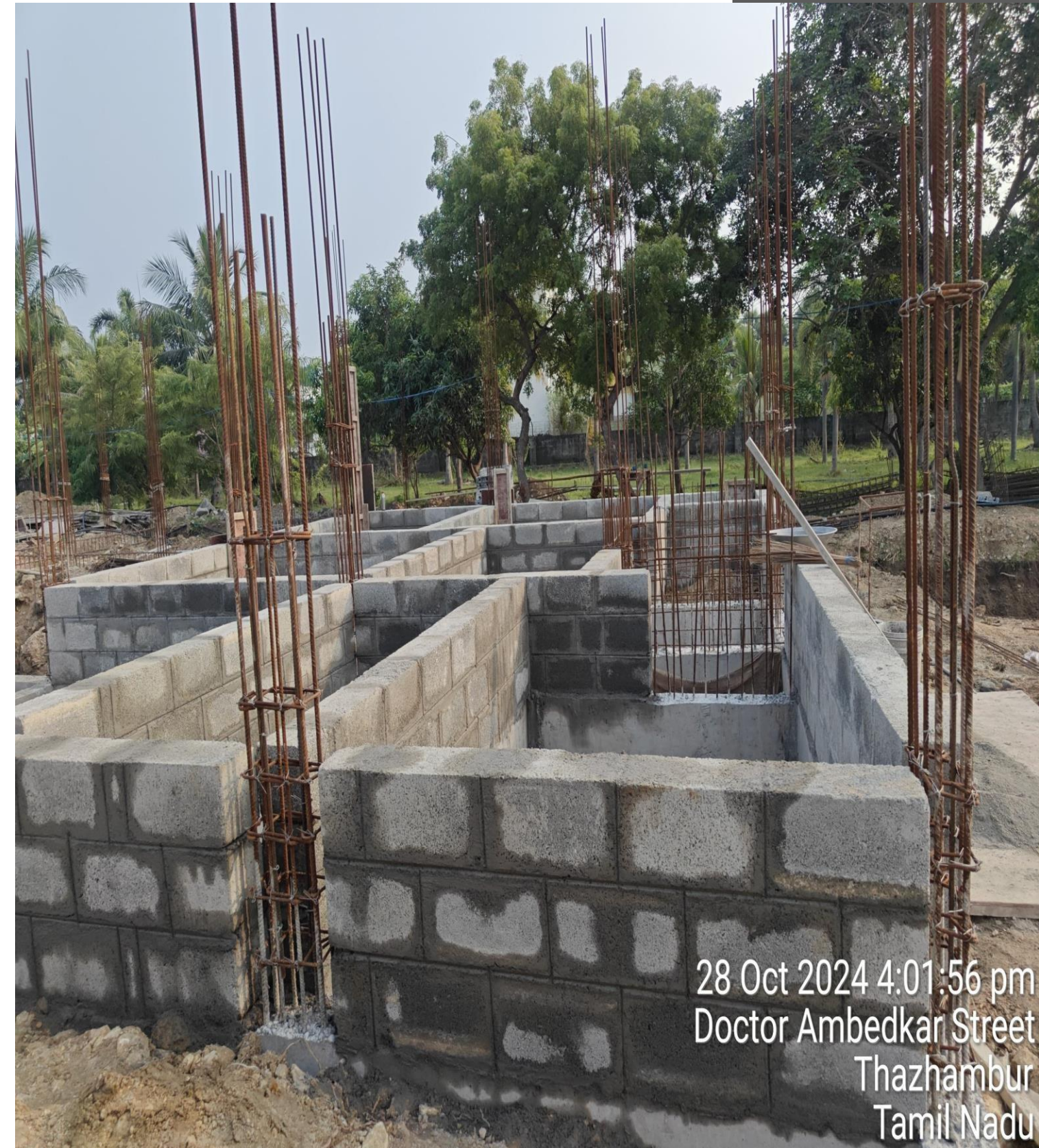
Villa No 6 and 11 Below GF level Block work in progress
