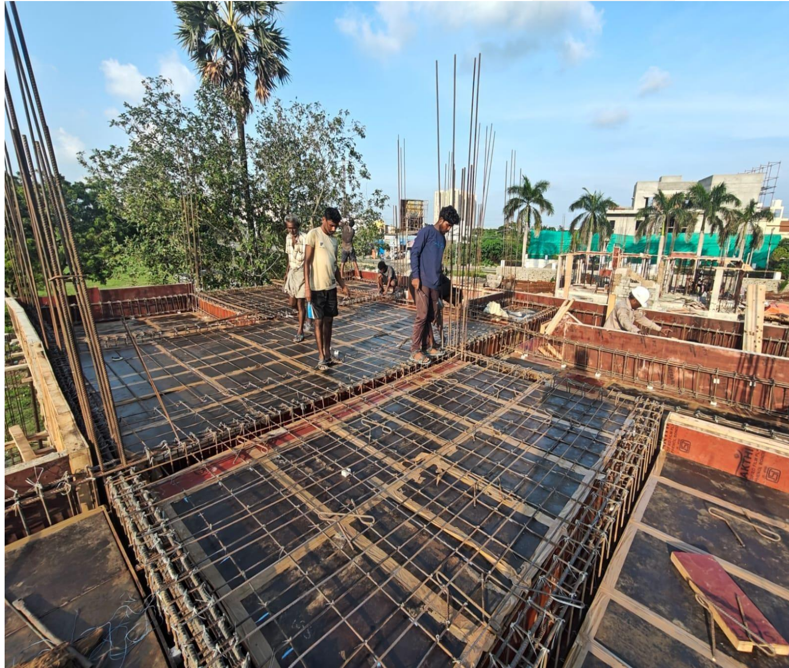
Villa No.16 GF Roof Slab Reinforcement & Electrical Conduit Pipe Laying work in Progress
