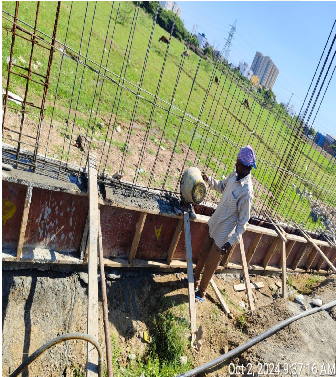
Compound wall - RCC Wall concrete work in Progress
