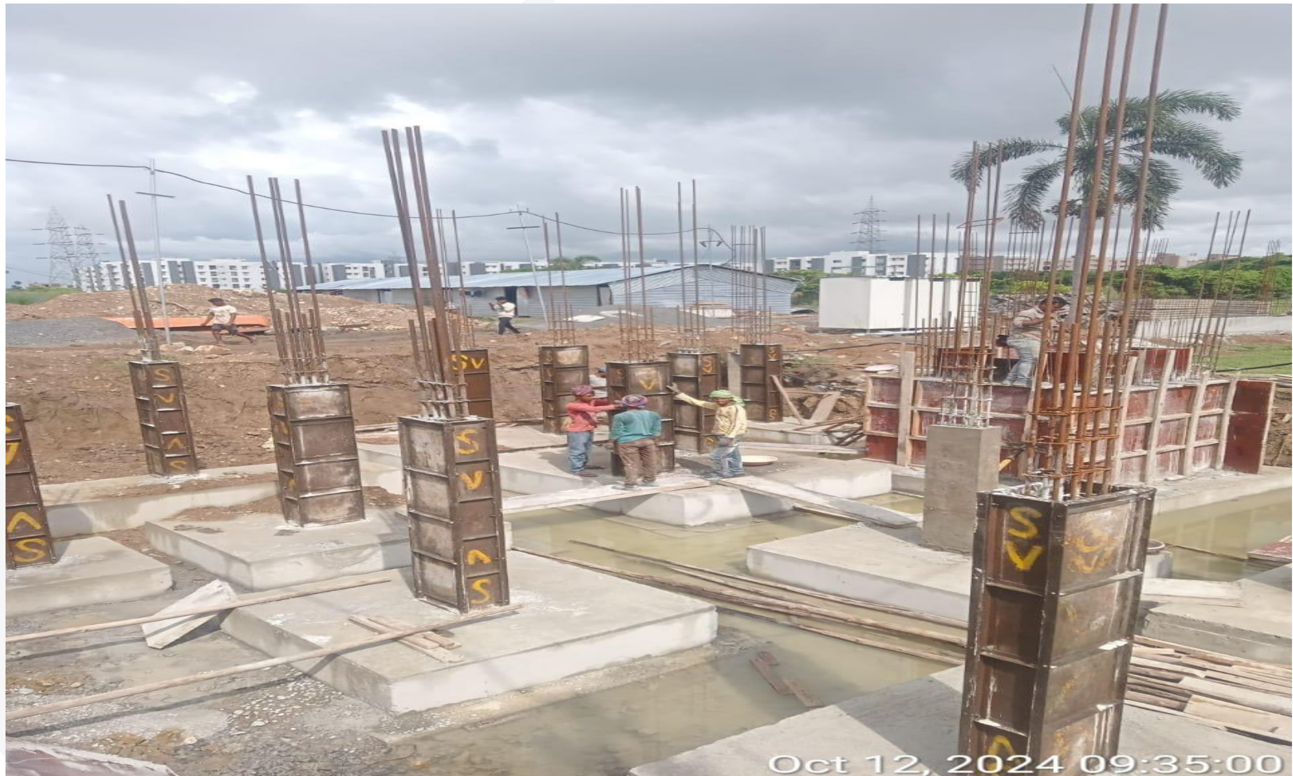
Villa No.12 Pedestal Column Shuttering & Concrete Completed
