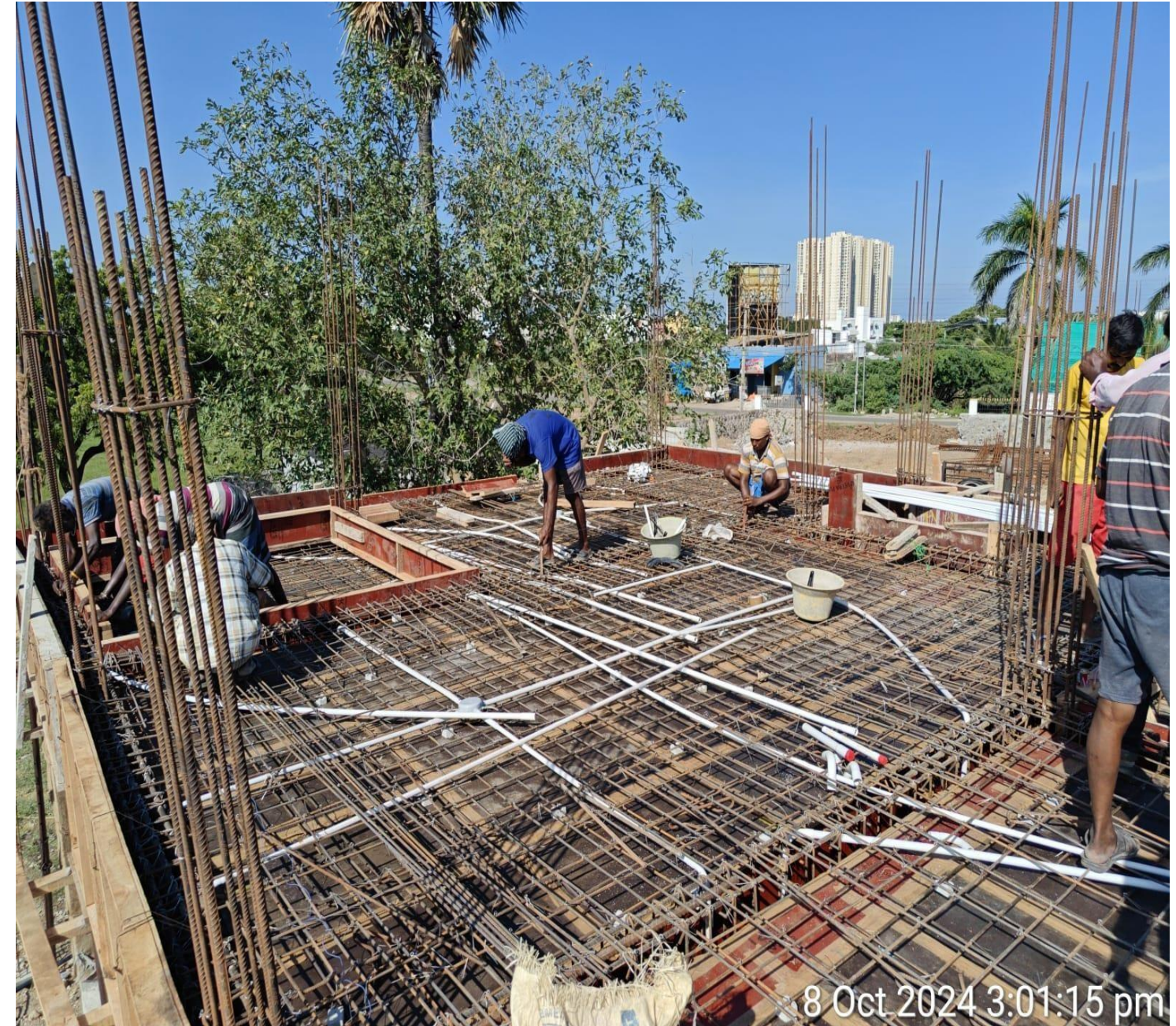
Villa No.16 GF Roof Slab Reinforcement & Electrical Conduit Pipe Laying work in Progress
