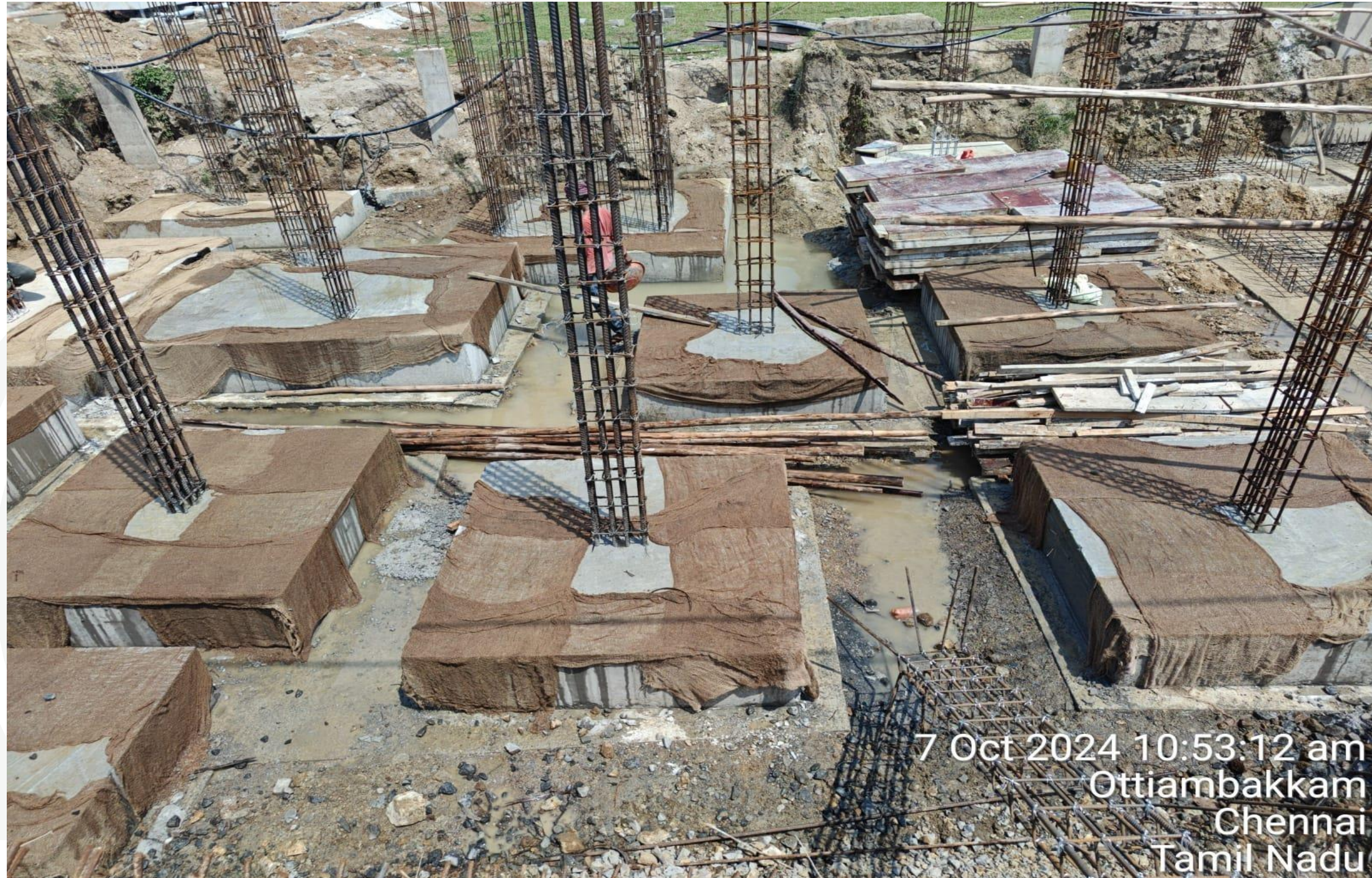
Villa No 12 Footing concrete completed
