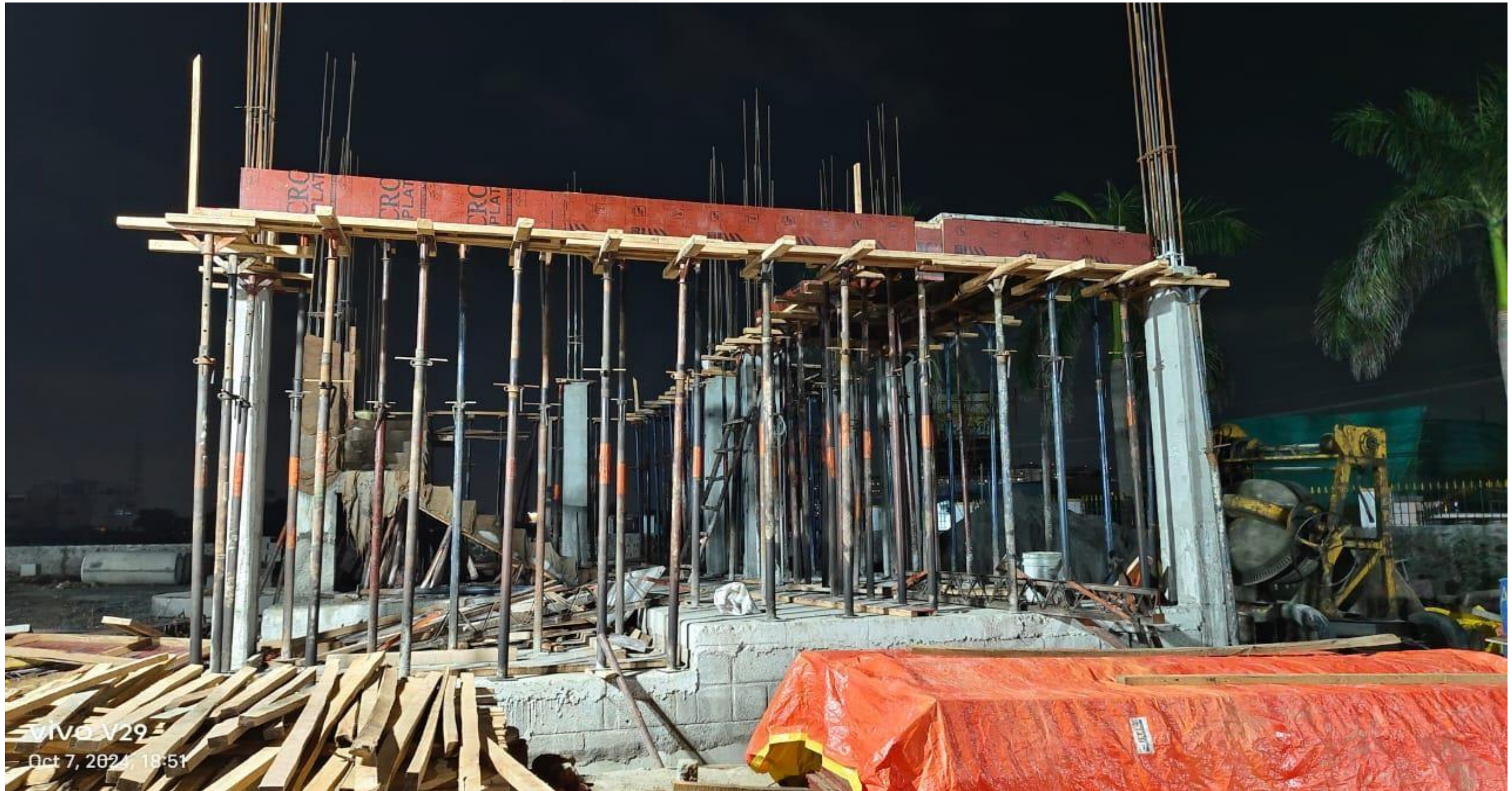
Villa No 20 GF Roof Slab Shuttering work in Progress
