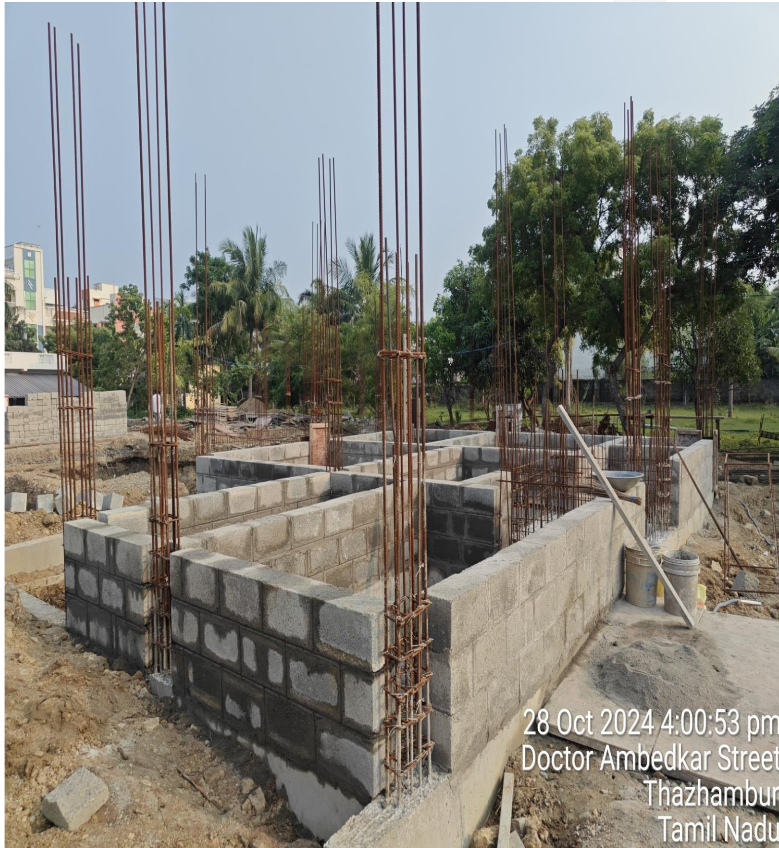
Villa No 6 and 11 Below GF level Block work in progress
