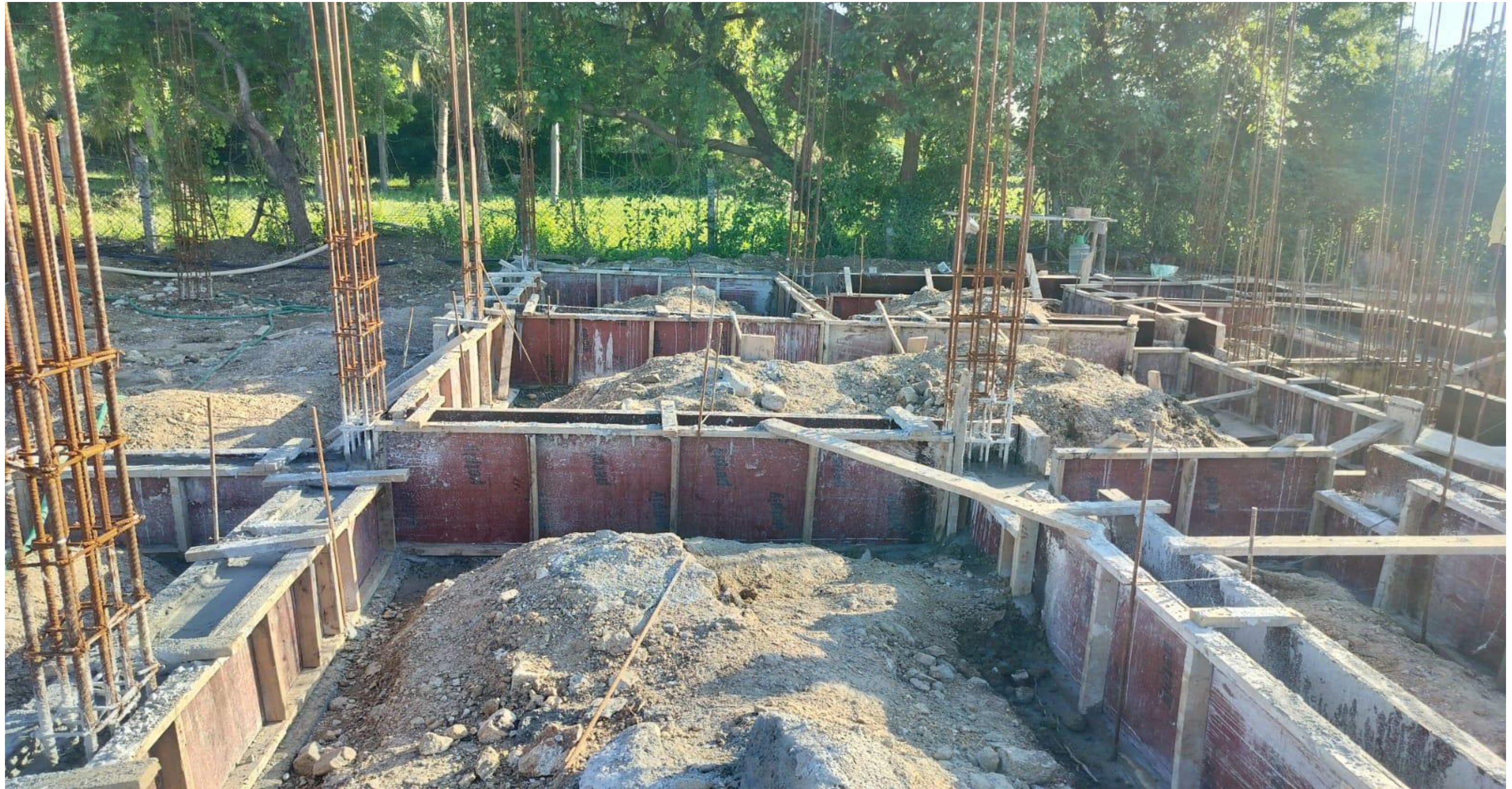
Villa no 11 Plinth beam concrete completed
