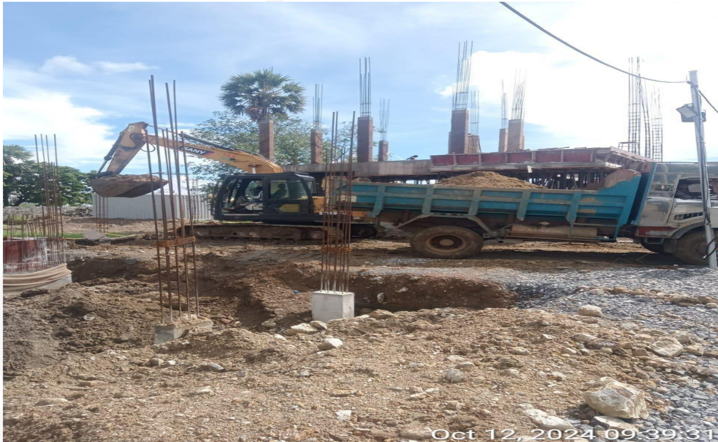
Villa no 15 Earth work Excavation in progress
