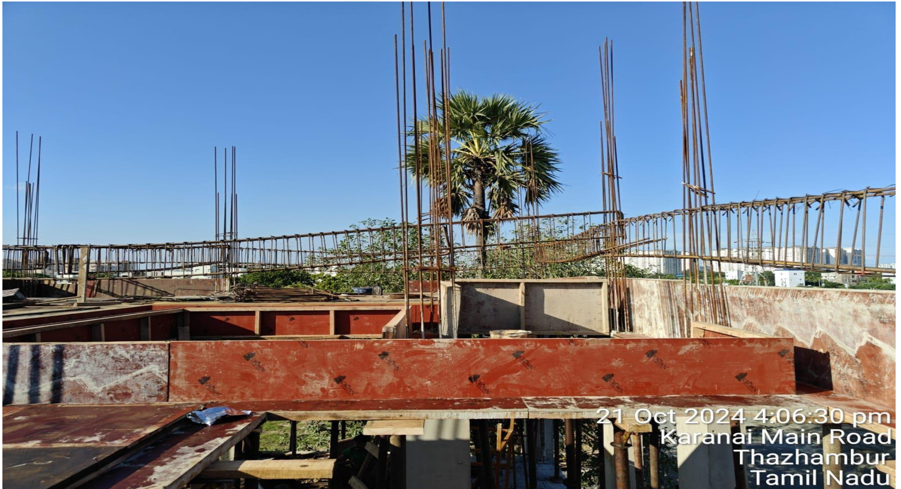
Villa No 16 FF Roof Slab shuttering and Reinforcement work in Progress
