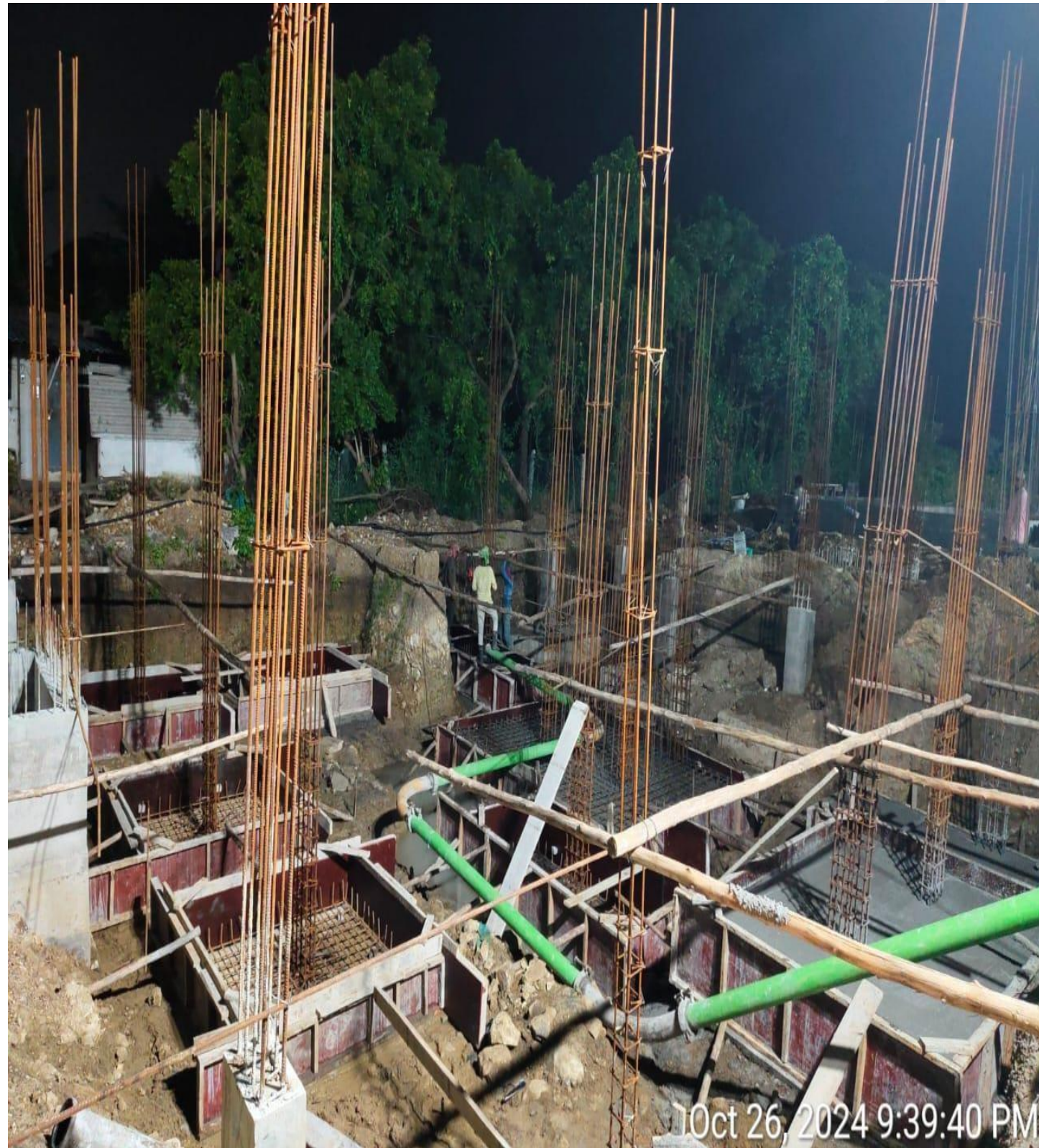
Villa no 9 All Footing Concrete Work Completed
