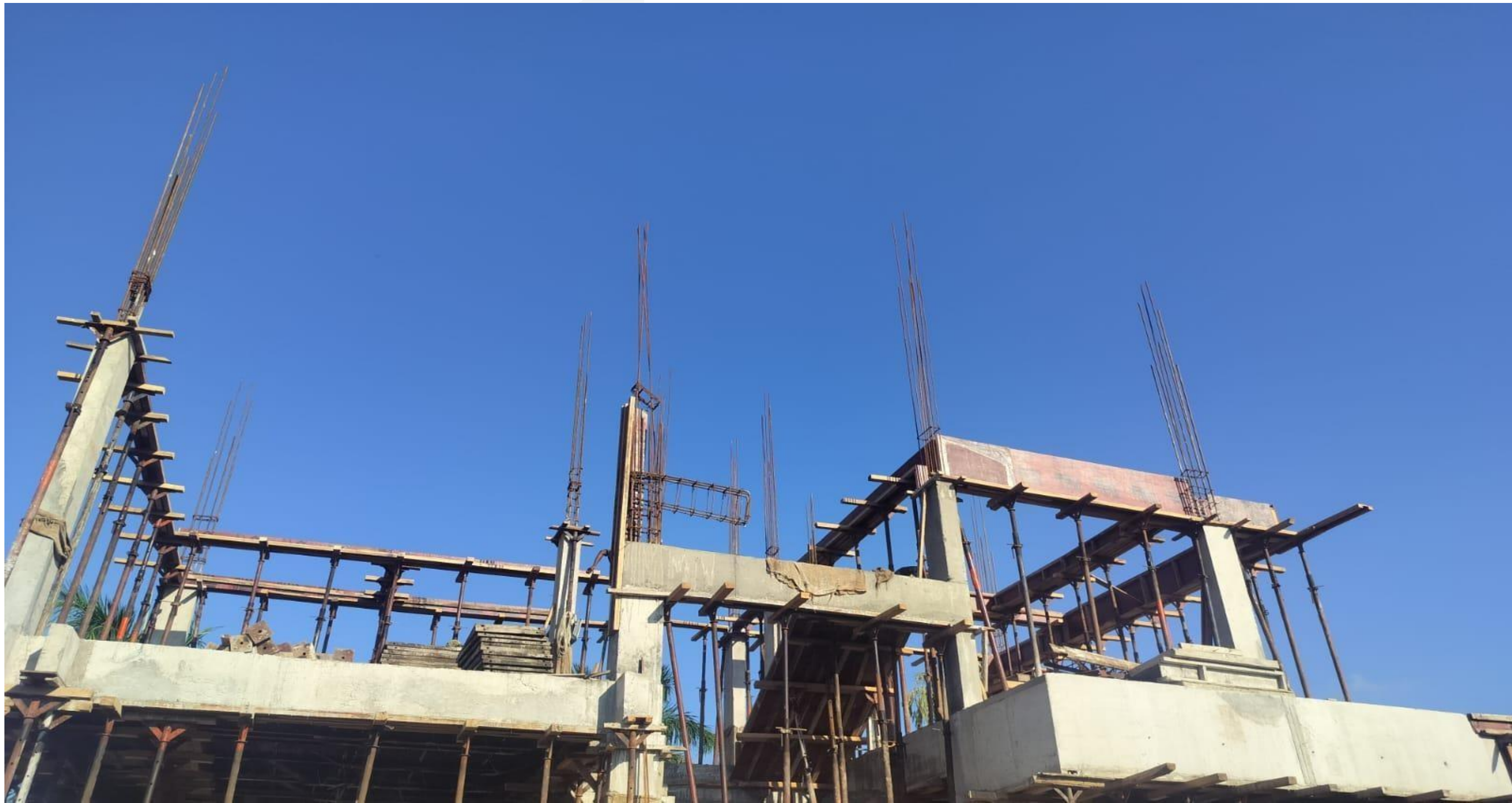
Villa No 20 FF Roof Slab shuttering work in Progress
