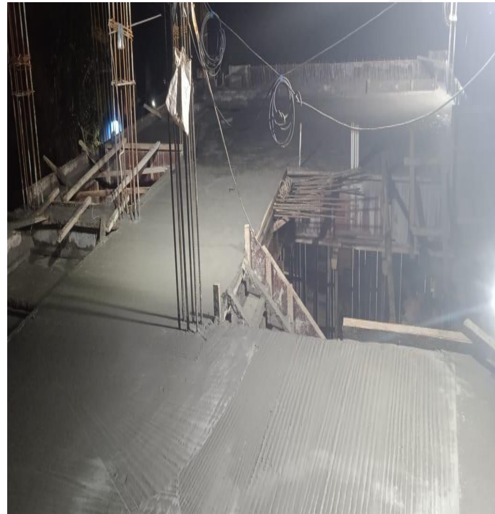
Villa No 20 FF Roof Concrete Completed
