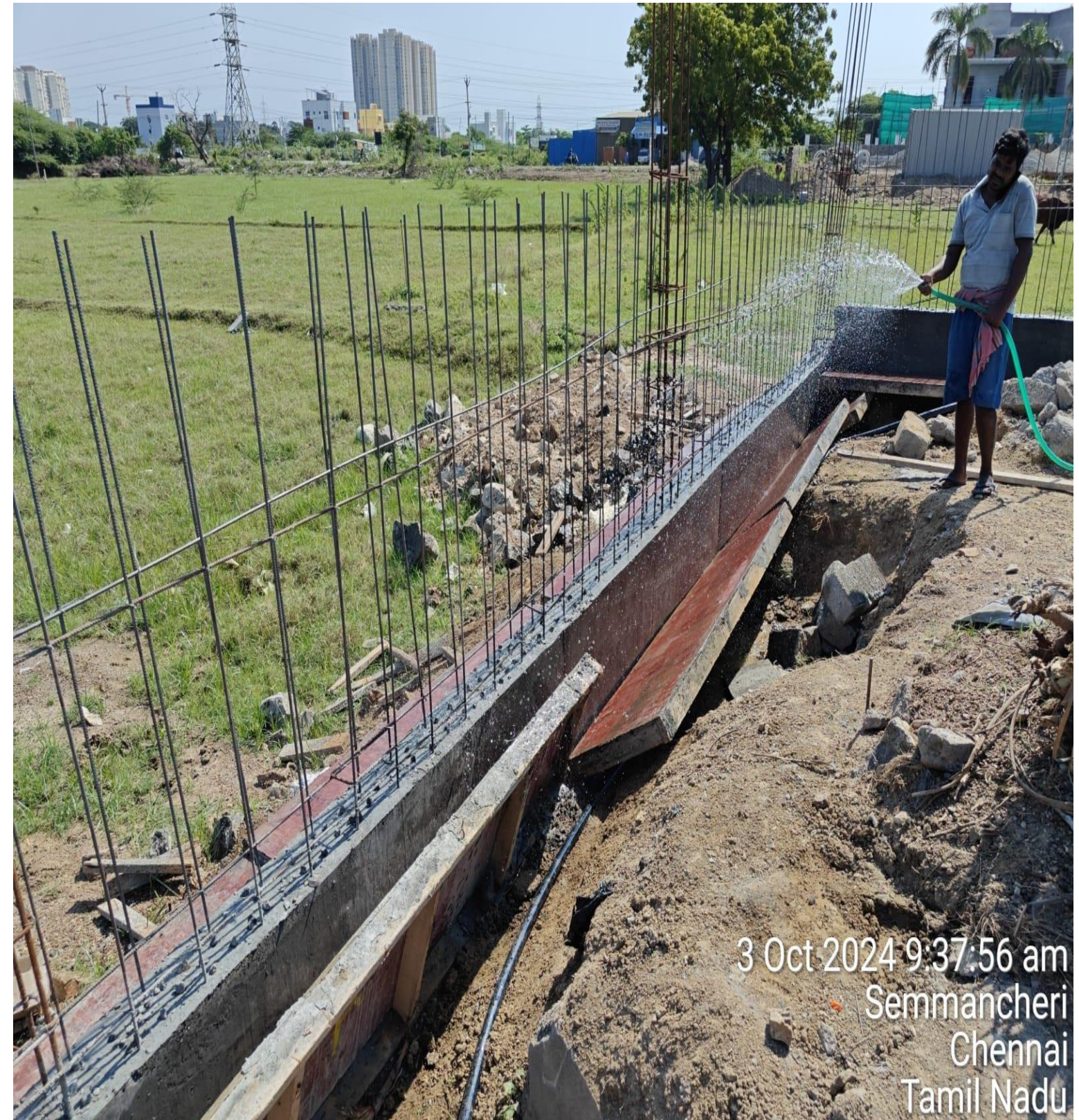
Compound wall - RCC Wall concrete work in Progress
