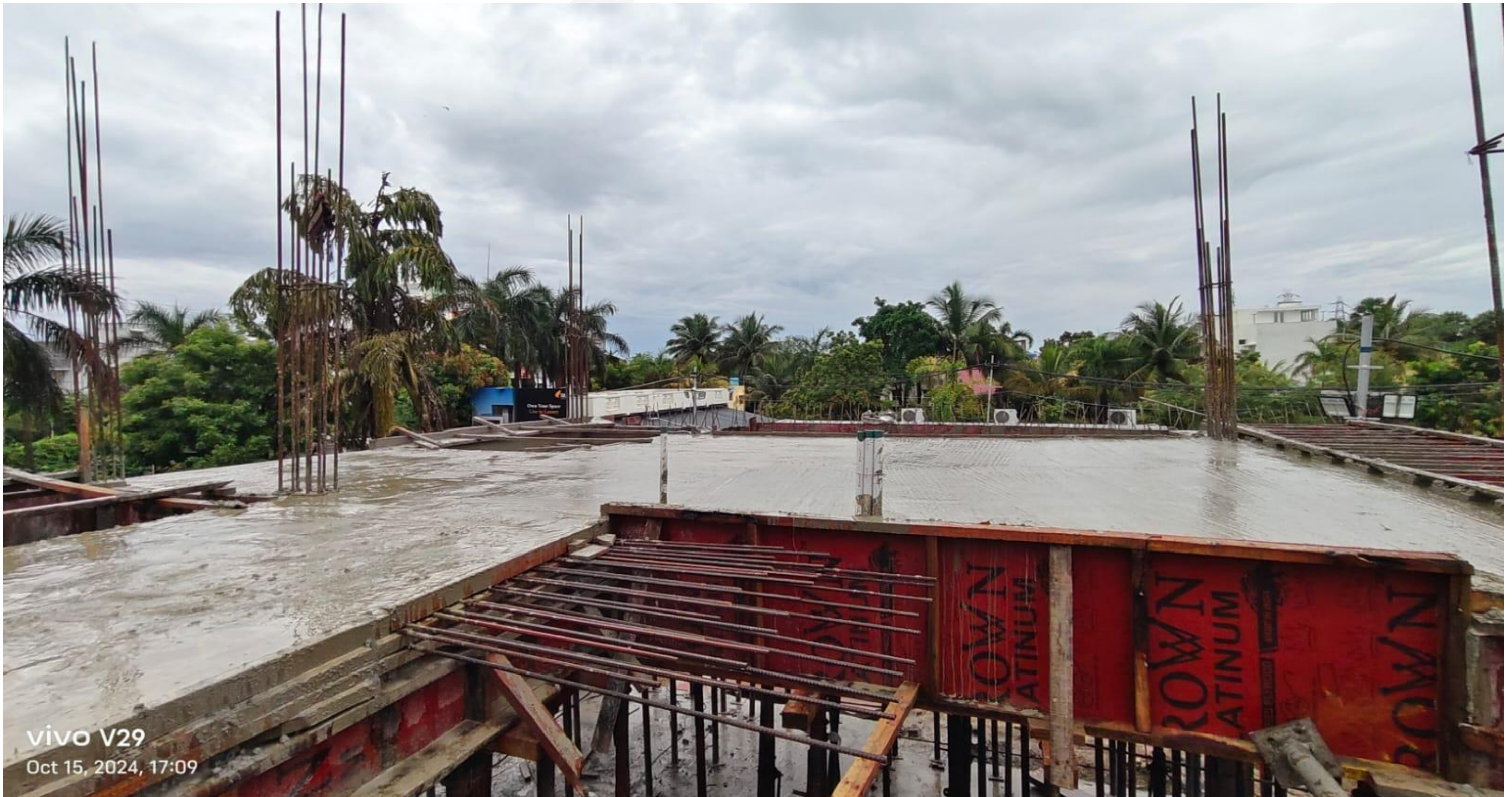
Villa No 20 GF Roof Slab Concrete Completed
