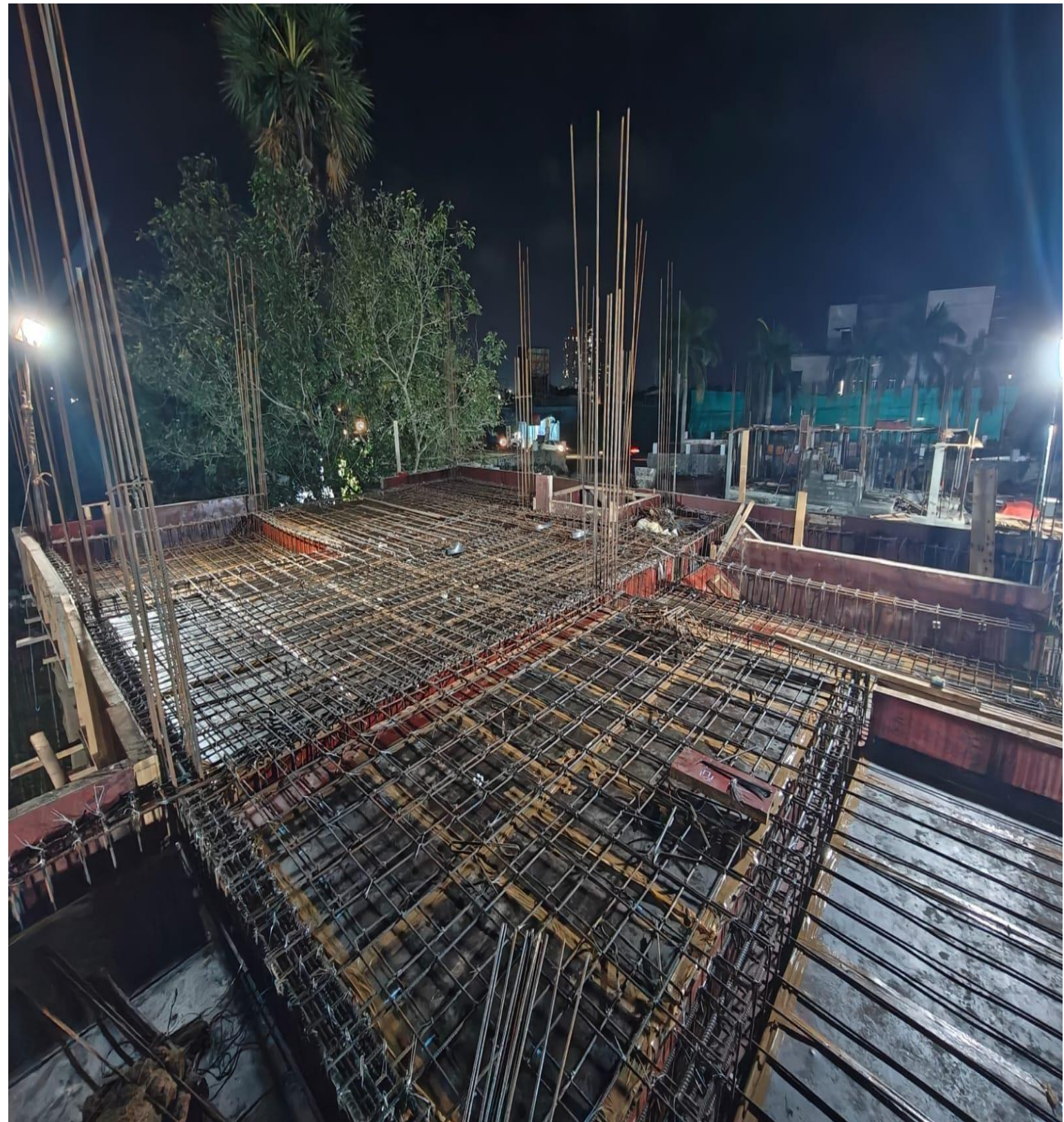
Villa No 16 GF Roof slab shuttering and Reinforcement work in progress
