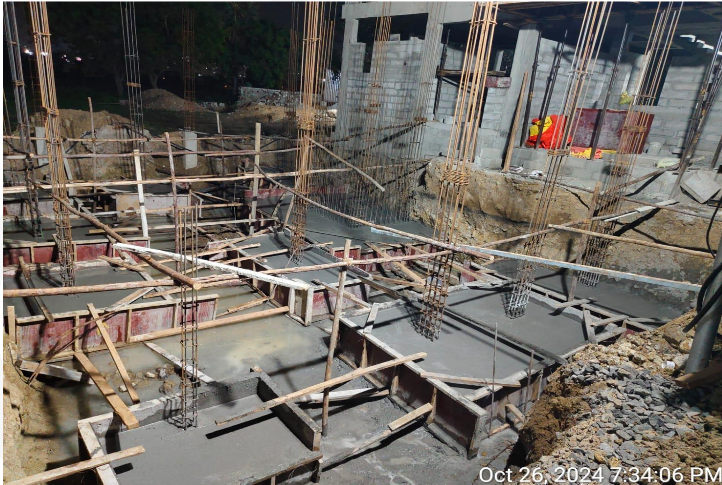
Villa No 15 All Footing Concrete Completed
