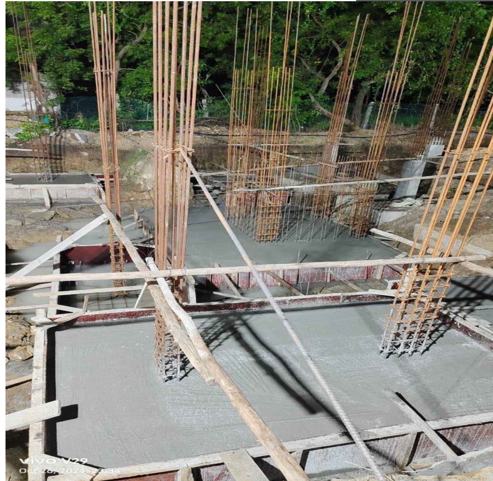
Villa no 9 All Footing Concrete Work Completed
