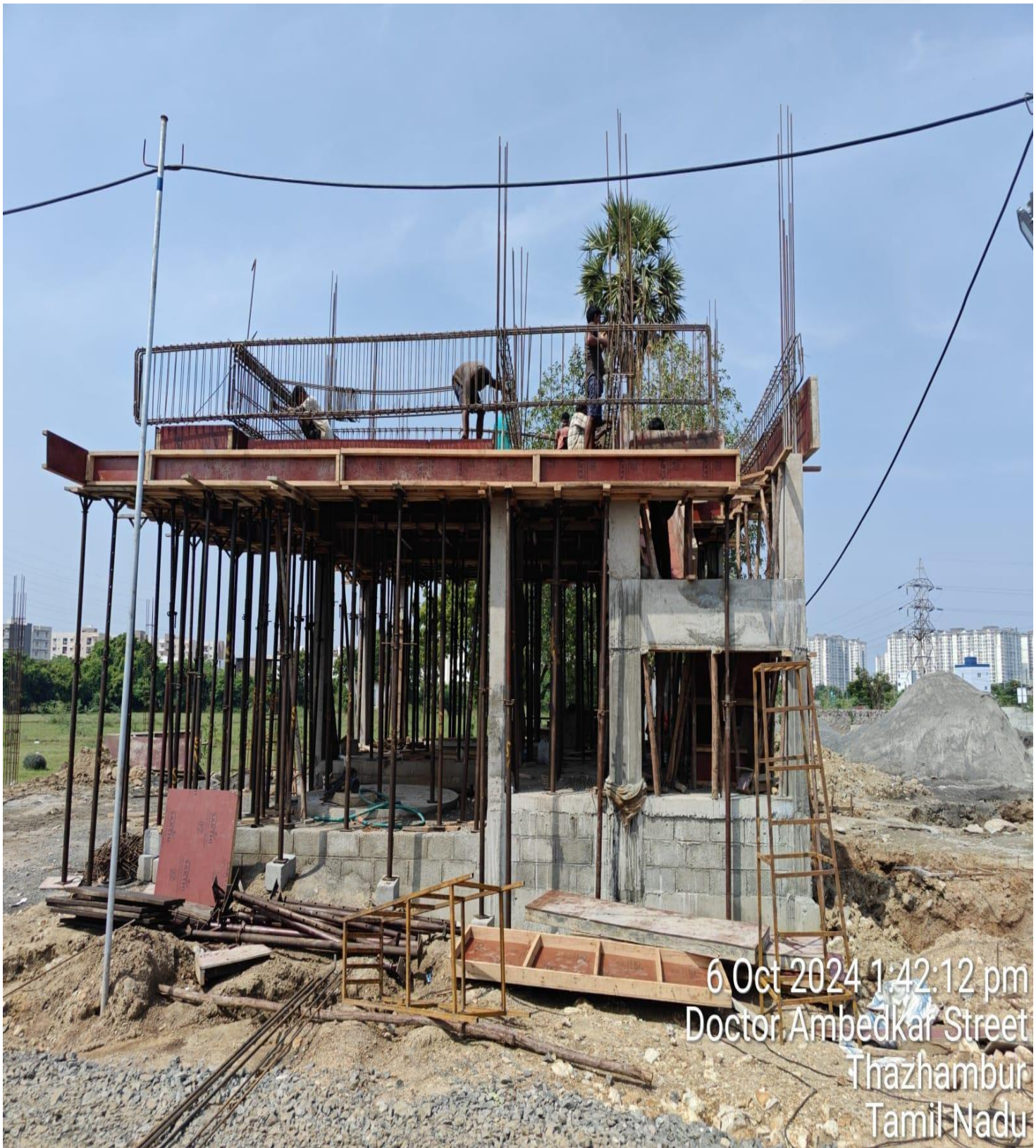
Villa No 16 GF Roof slab shuttering and Reinforcement work in progress
