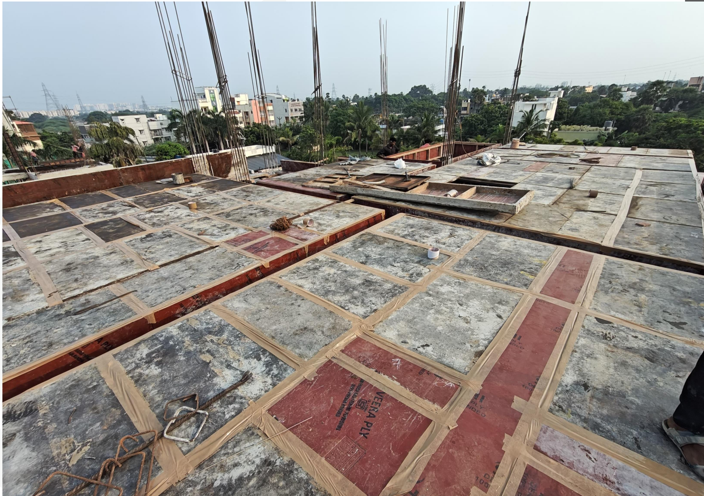
Villa No 16 Terrace Floor slab shuttering work in progress
