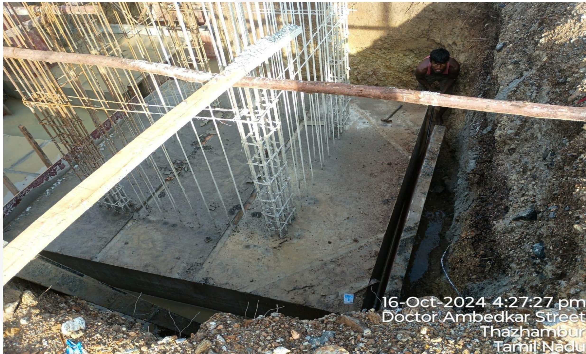
Villa no 17 Footing concrete work completed
