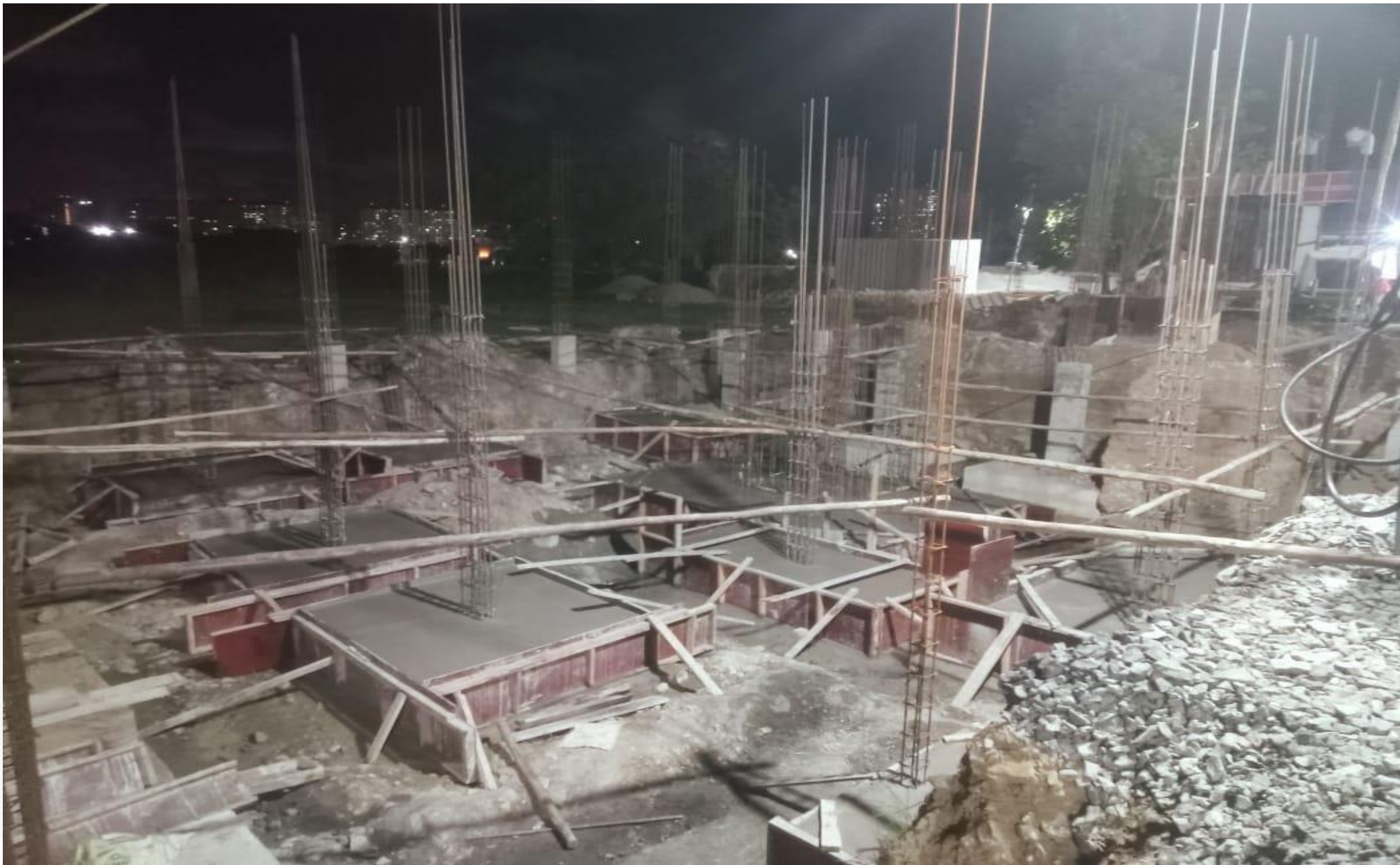
Villa No.13 Footing concrete completed
