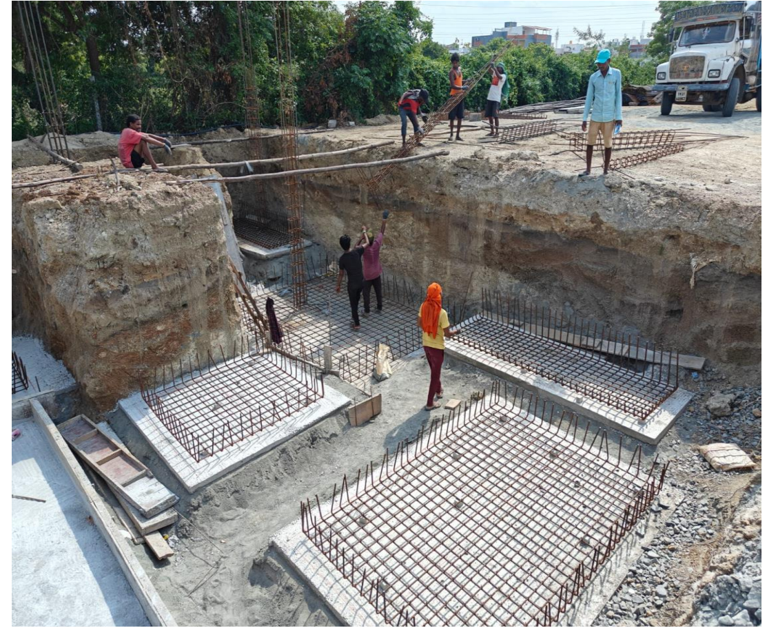
Villa No.11 Footing Reinforcement Steel
