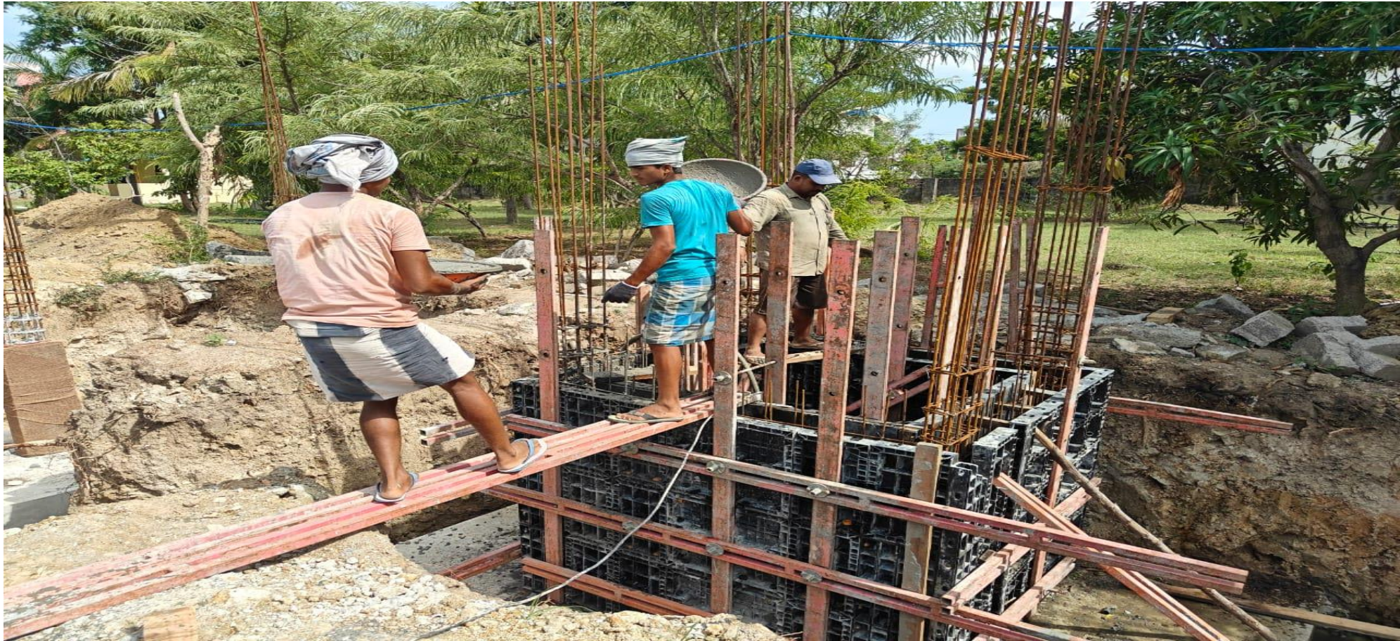
Villa No.04 Lift wall concrete work
