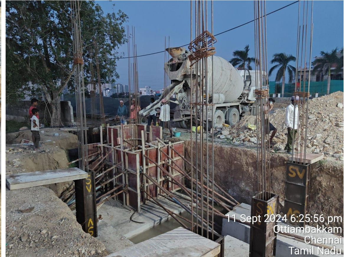
Villa No.16 Pedestal column Shuttering & Concrete
