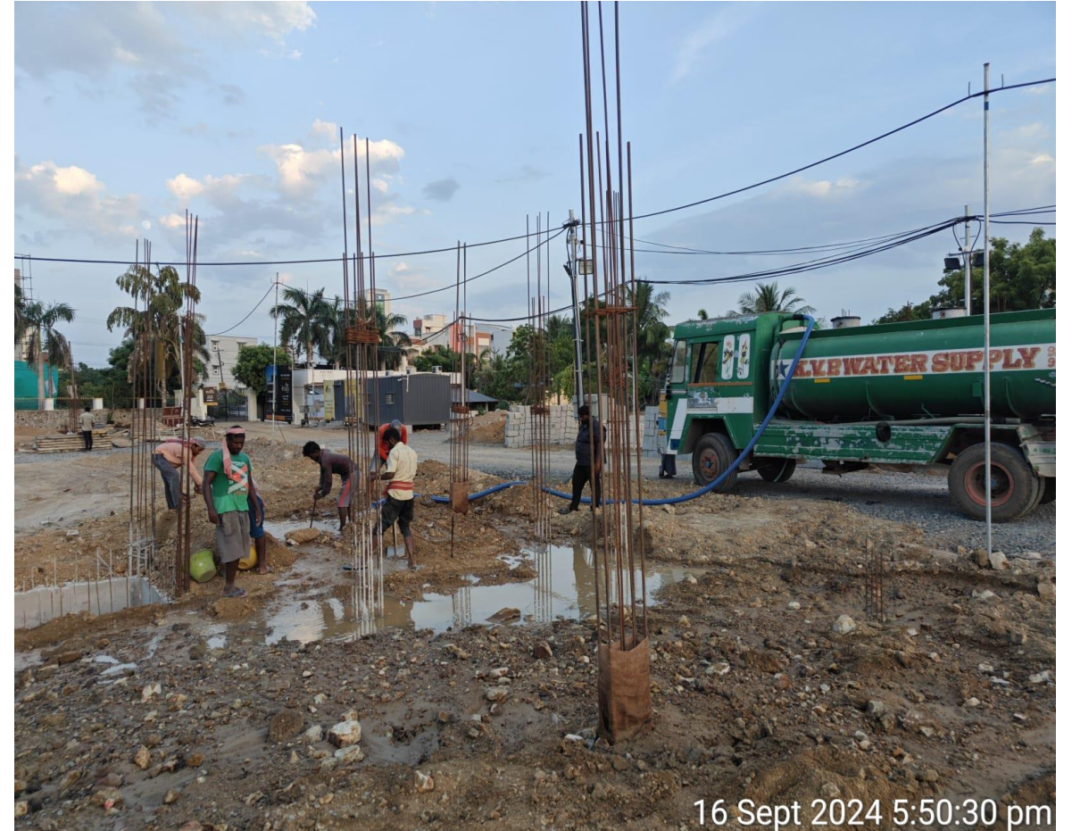
Villa No.16 Footing de shuttering & Pedestal column starter marking
