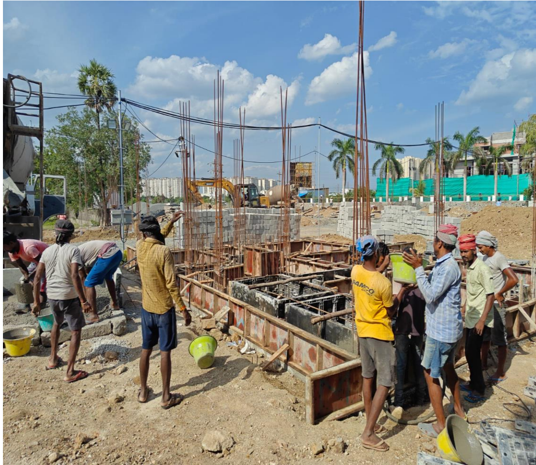
Villa No.06 Plinth beam Concrete
