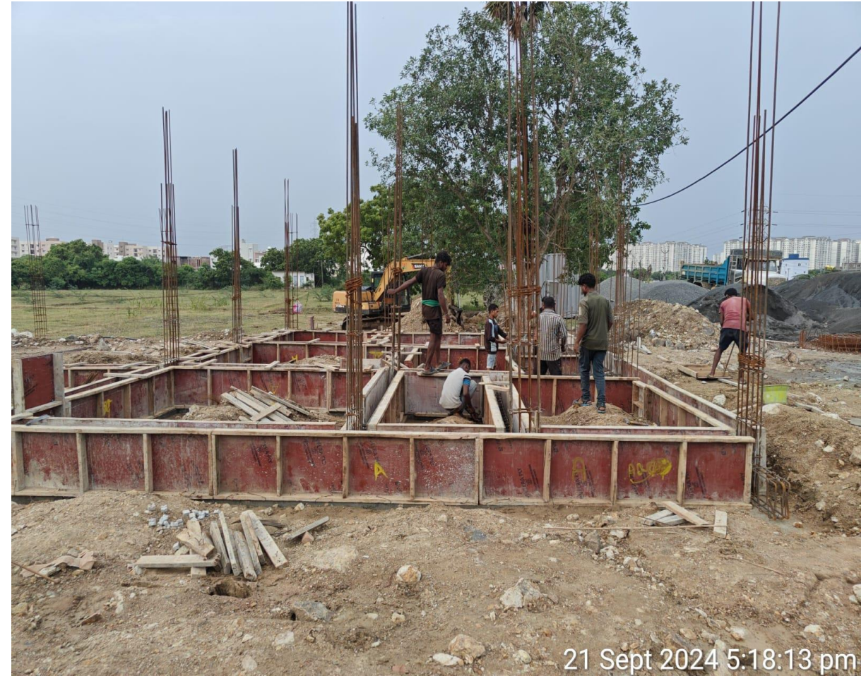
Villa No.16 Plinth Beam Shuttering
