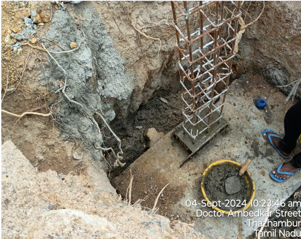
Compound wall Pedestal column starter concrete & shuttering
