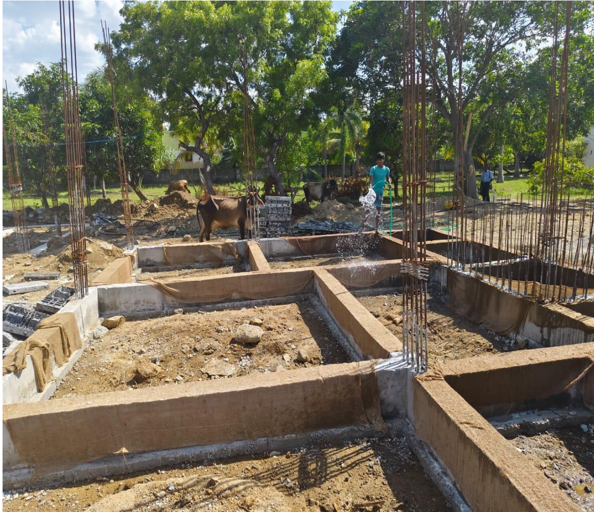
Villa No.06 Plinth beam Concrete
