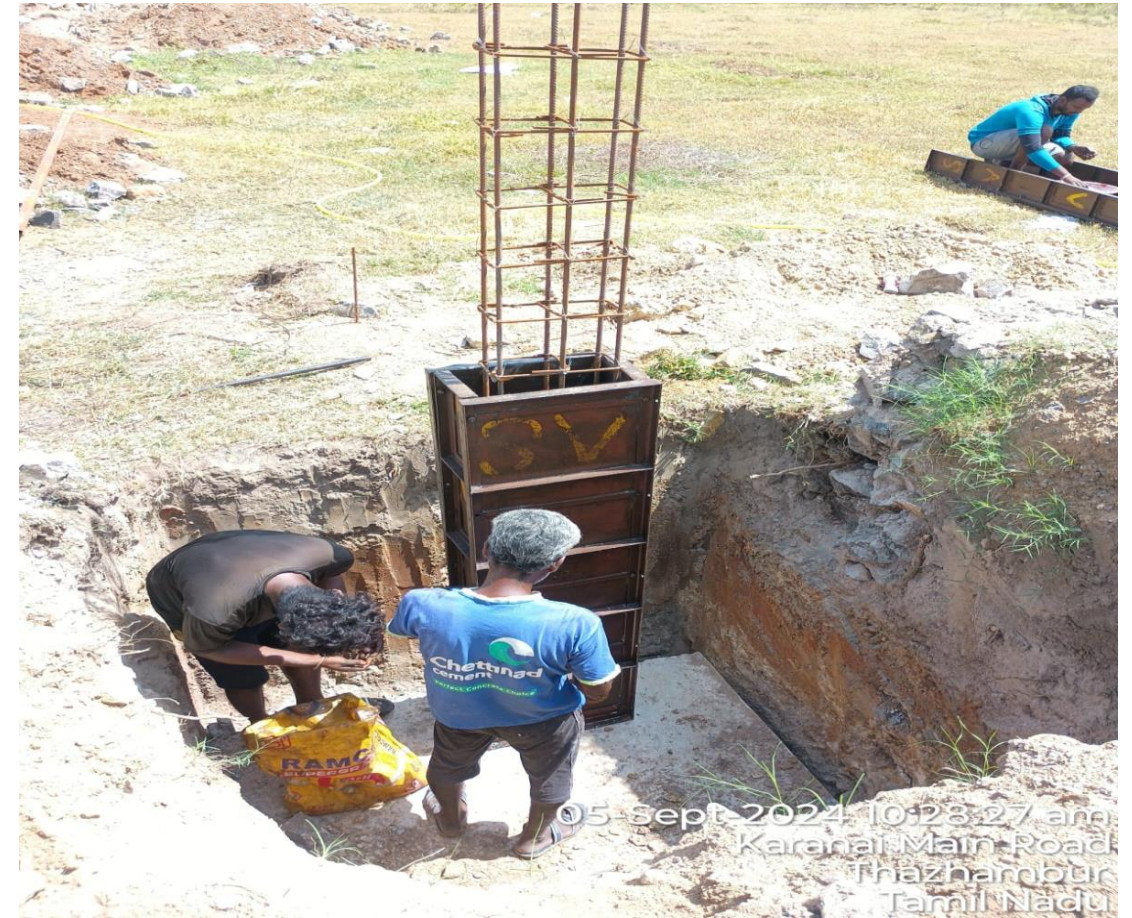
Compound wall Pedestal column starter concrete & shuttering
