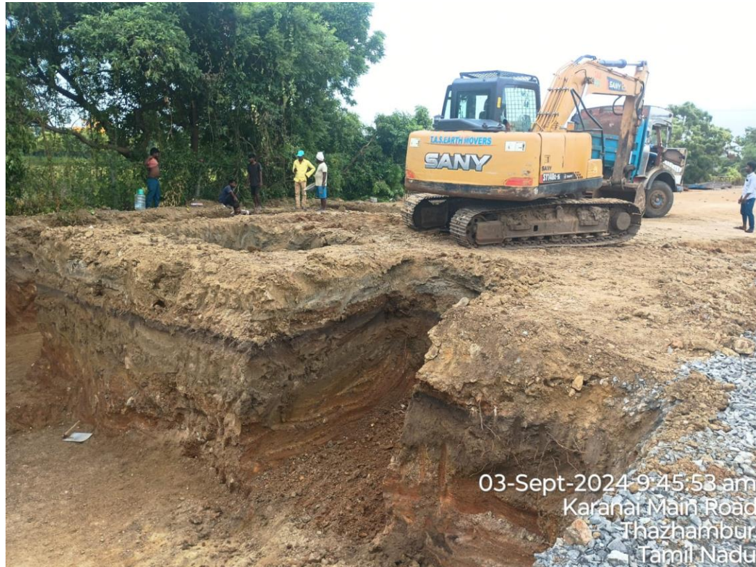
Villa No.11 Footing Earthwork excavation & Quarry dust filling work
