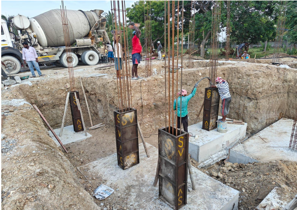
Villa No.08 Footing Reinforcement steel & Concrete
