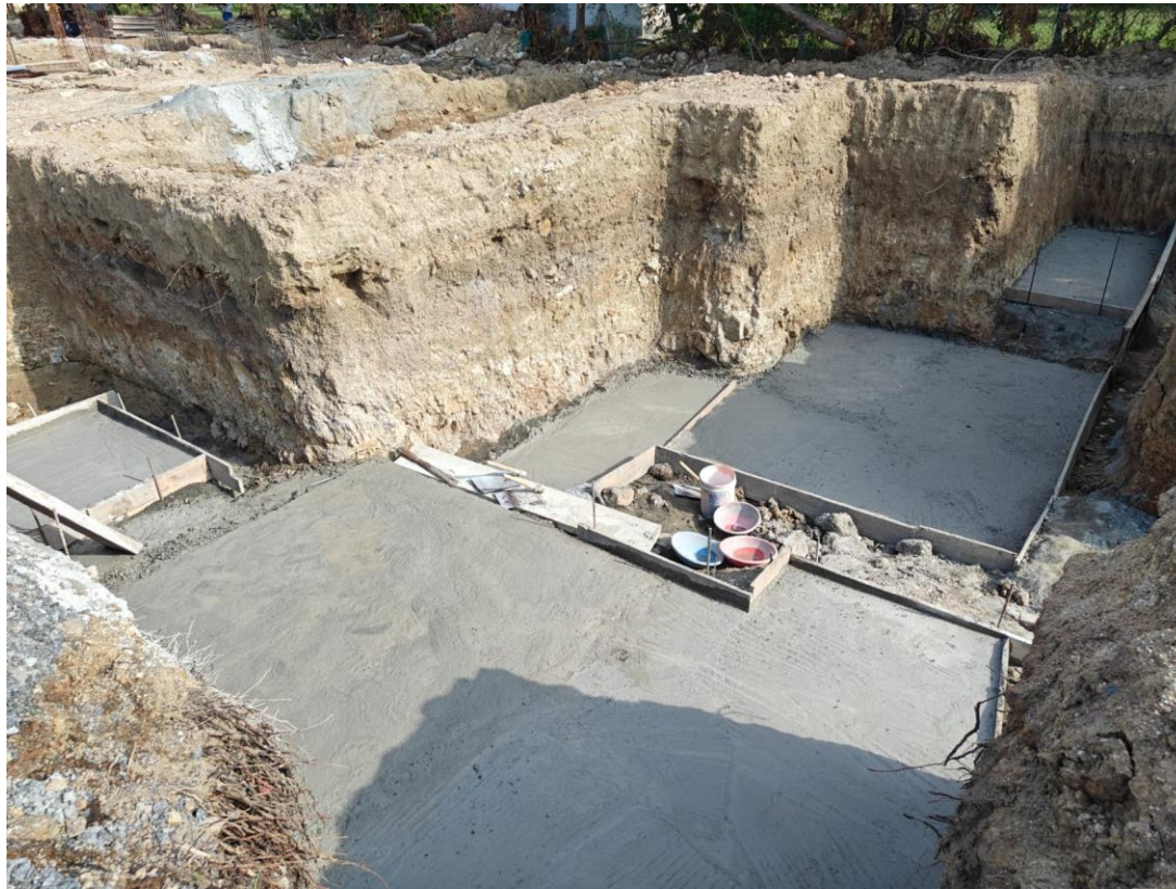
Villa No.10 Footing PCC & Reinforcement Steel
