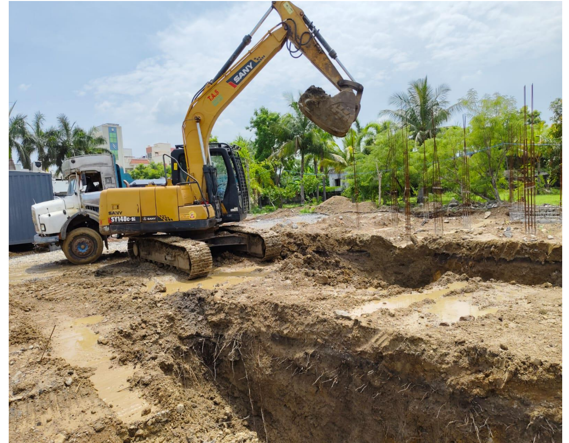
Villa No.05 Footing Earthwork Excavation
