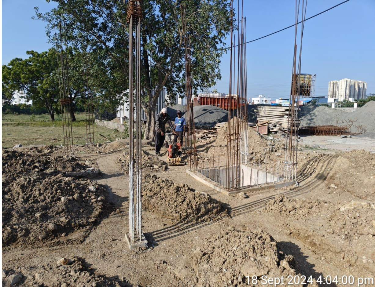
Villa No.16 Plinth beam Bottom soil compaction
