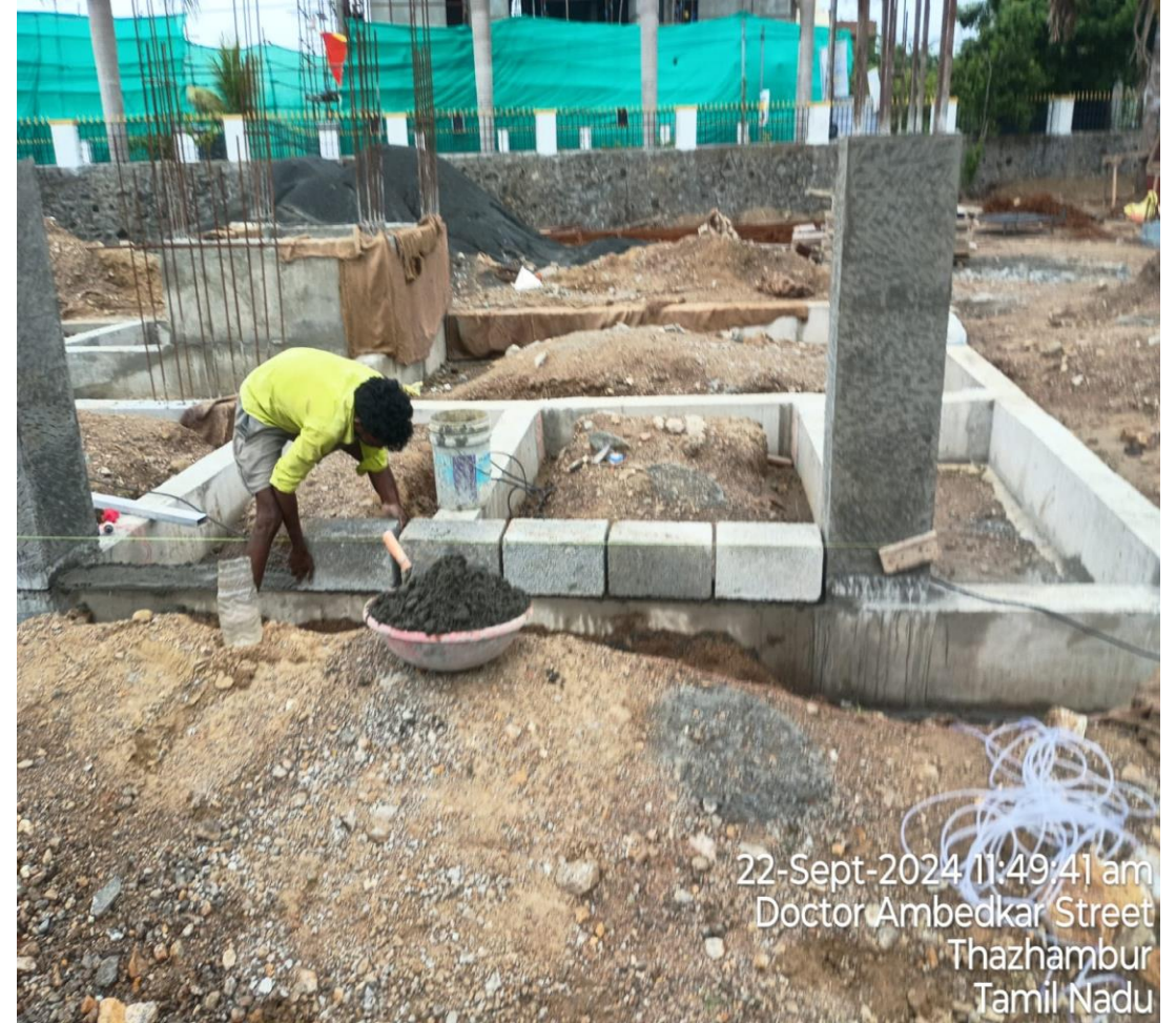
Villa No.20 Basement column Shuttering & concrete Block work
