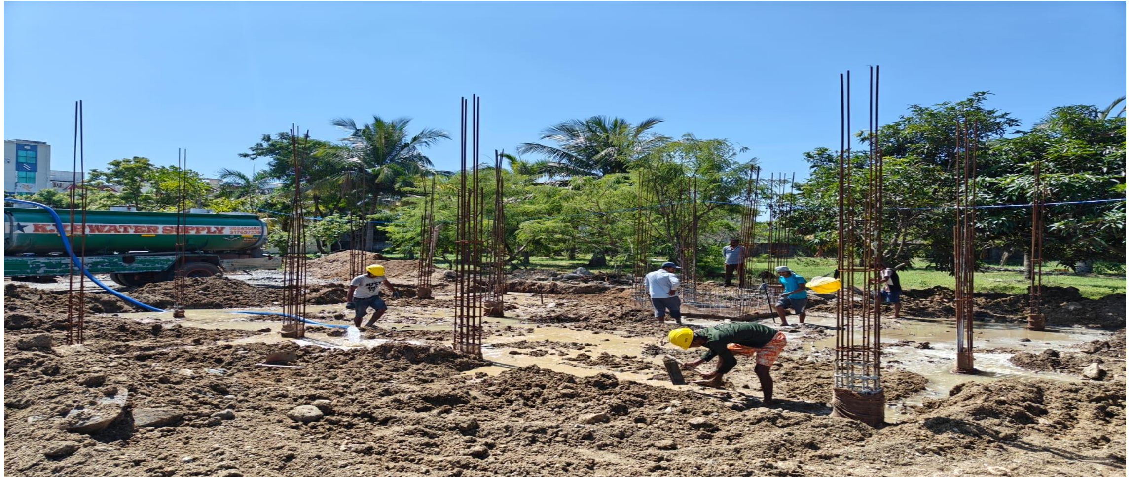
Villa No.04 Soil consolidation
