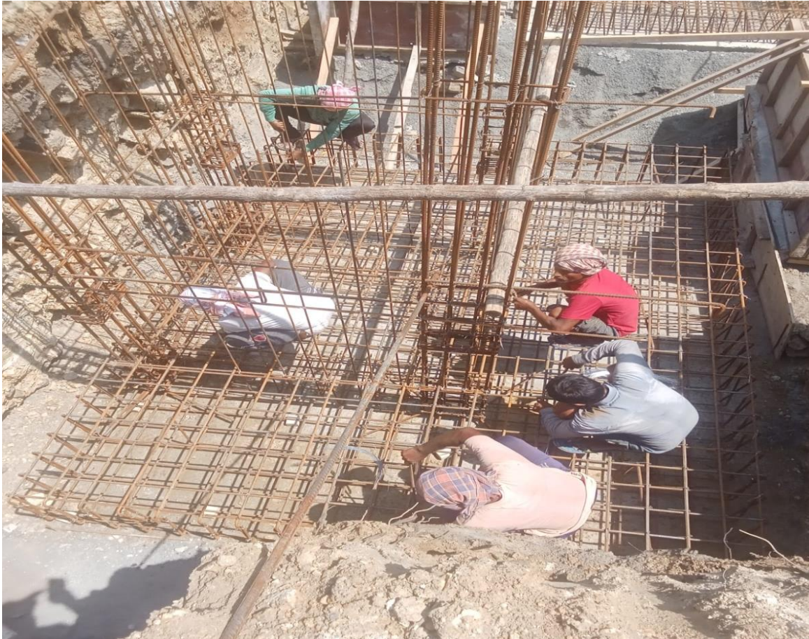
Villa No.08 Footing Reinforcement steel & Concrete
