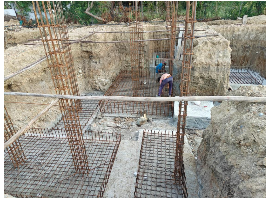
Villa No.10 Footing PCC & Reinforcement Steel
