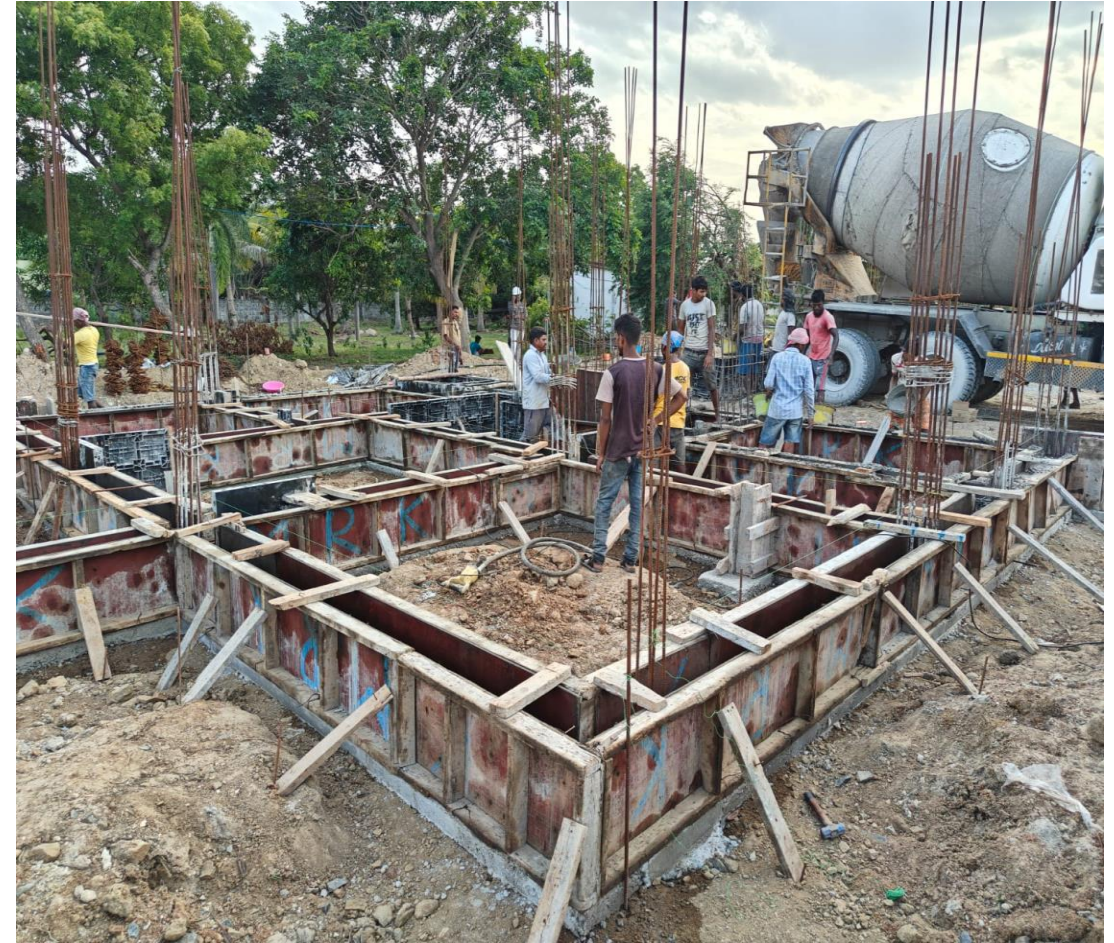
Villa No.06 Plinth beam Concrete
