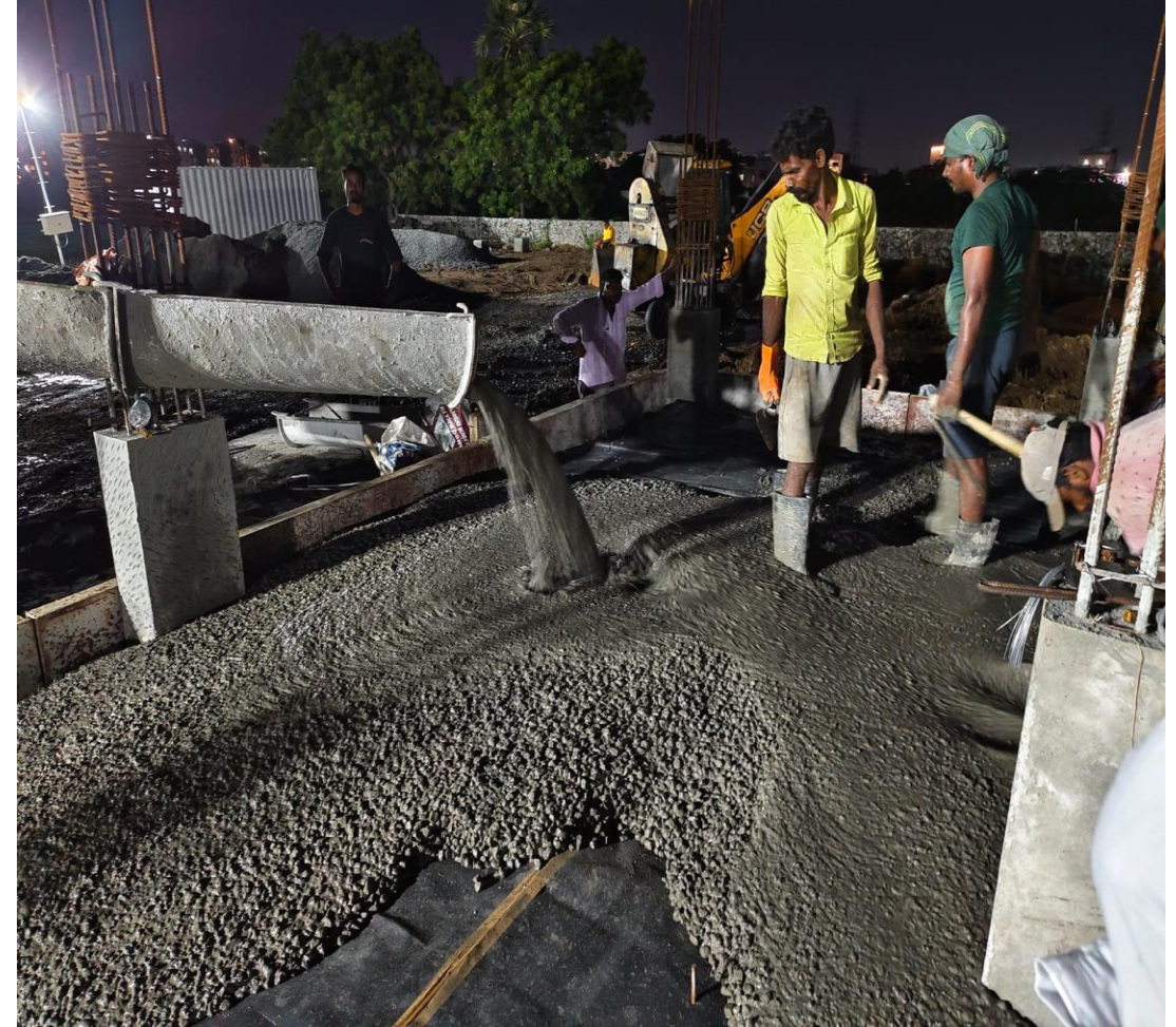
Villa No.20 GF PCC
