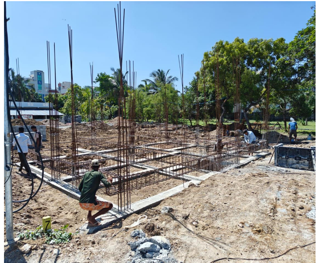
Villa No.06 Plinth beam Reinforcement
