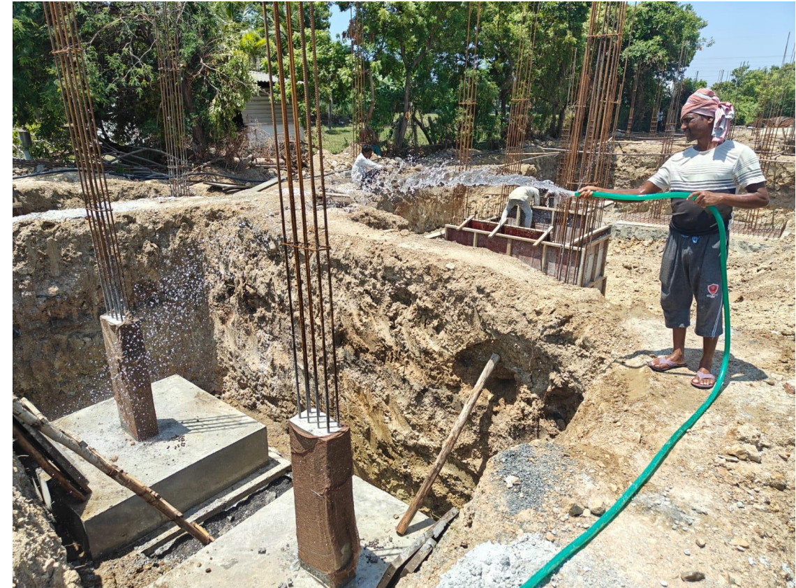
Villa No.08 Footing Reinforcement steel & Concrete
