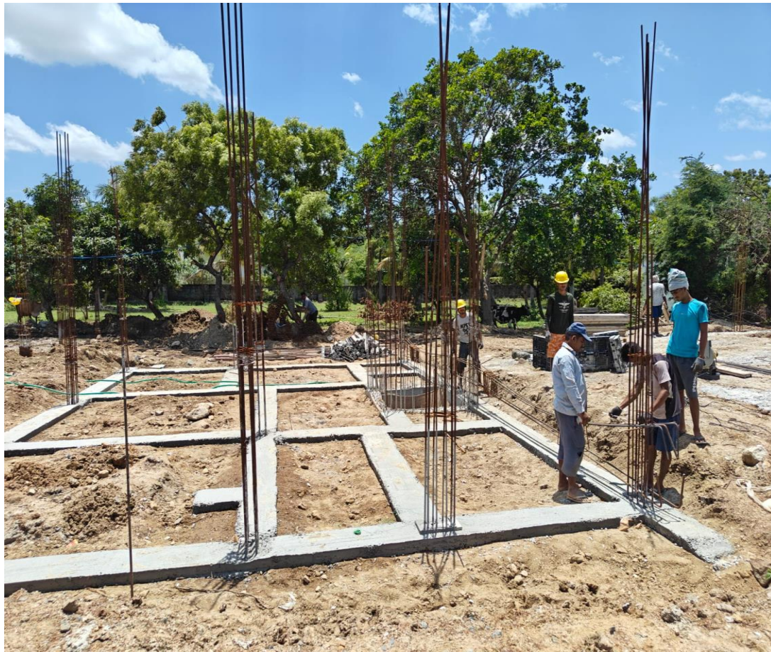
Villa No.06 Plinth beam Reinforcement
