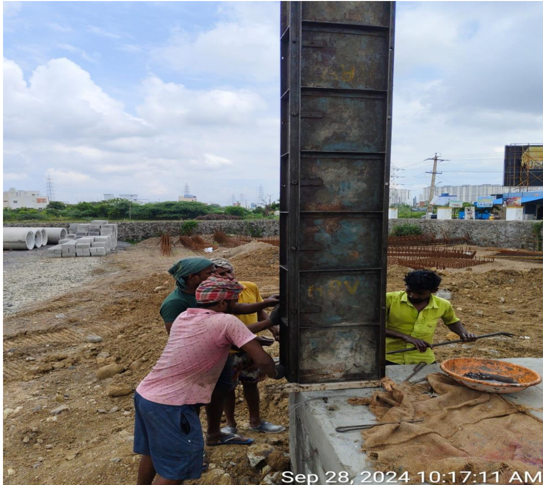
Villa No.20 GF Column shuttering & concrete
