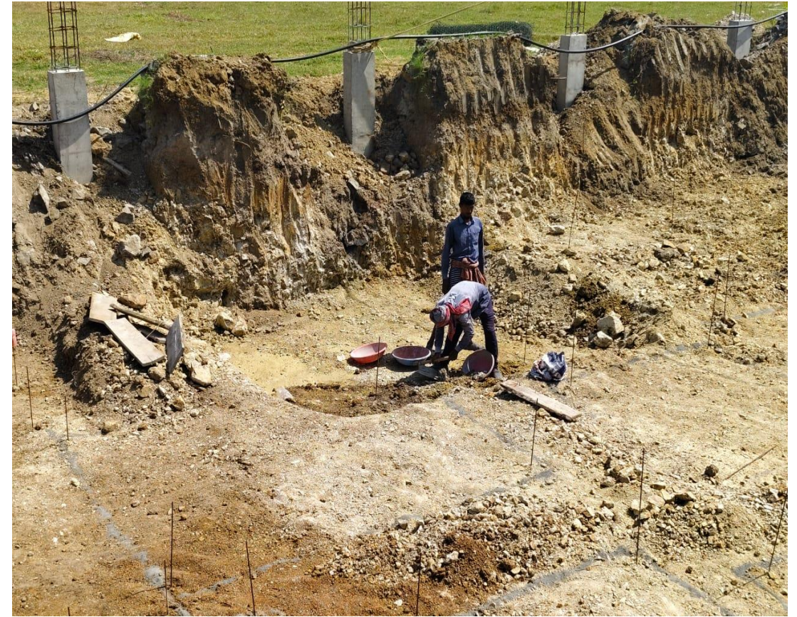
Villa No.12 Earthwork Excavation and Footing Dressing
