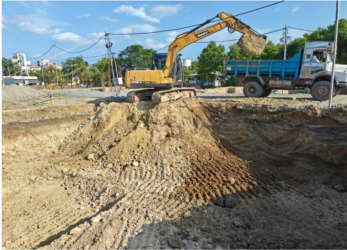
Villa No.12 Earthwork Excavation and Footing Dressing
