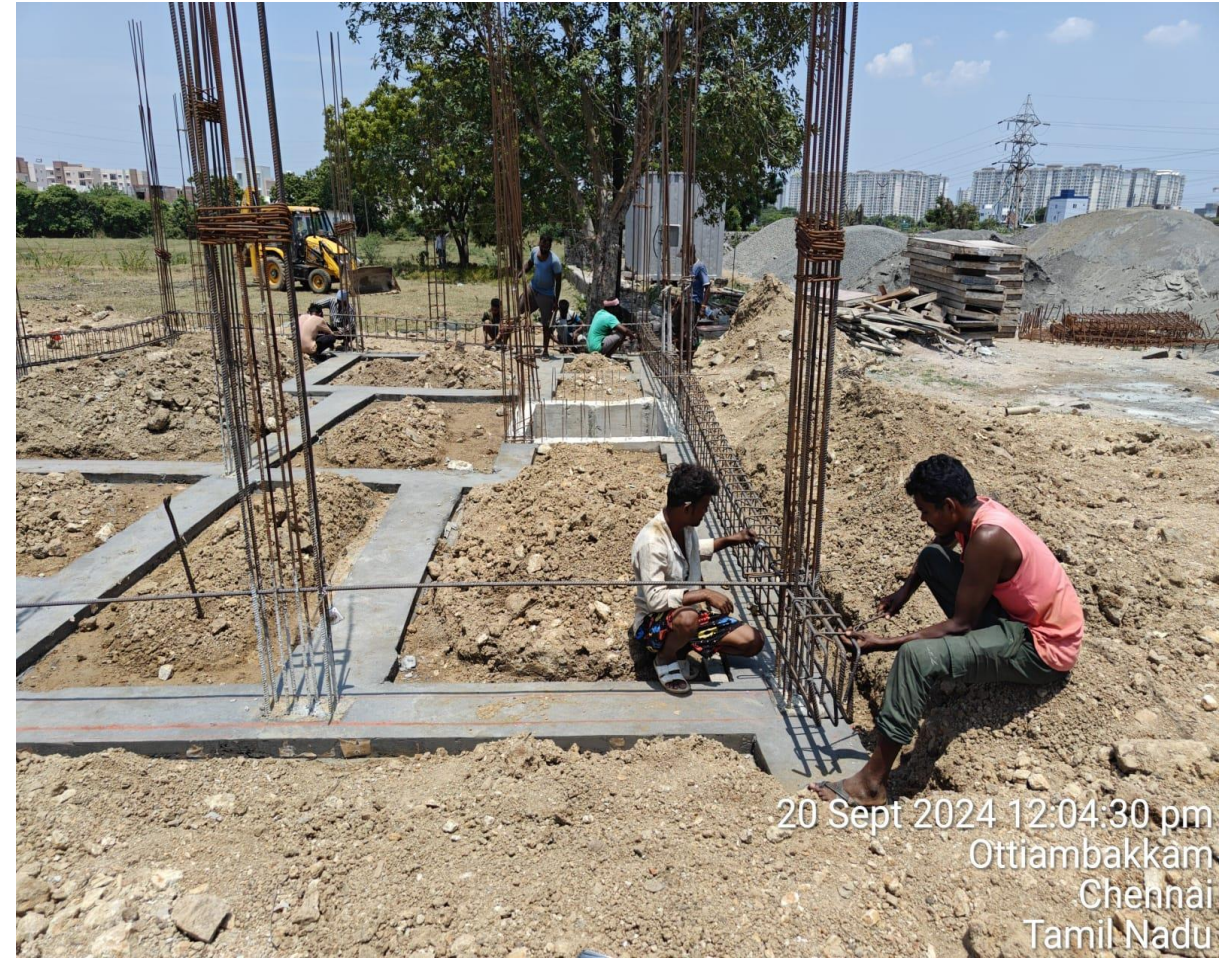
Villa No.16 Plinth Beam Reinforcement steel
