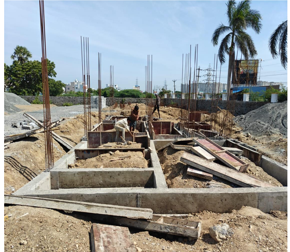
Villa No.20 Plinth Beam Concrete & Deshuttering
