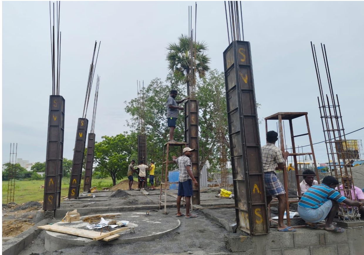
Villa No.16 GF Column Shuttering & Concrete
