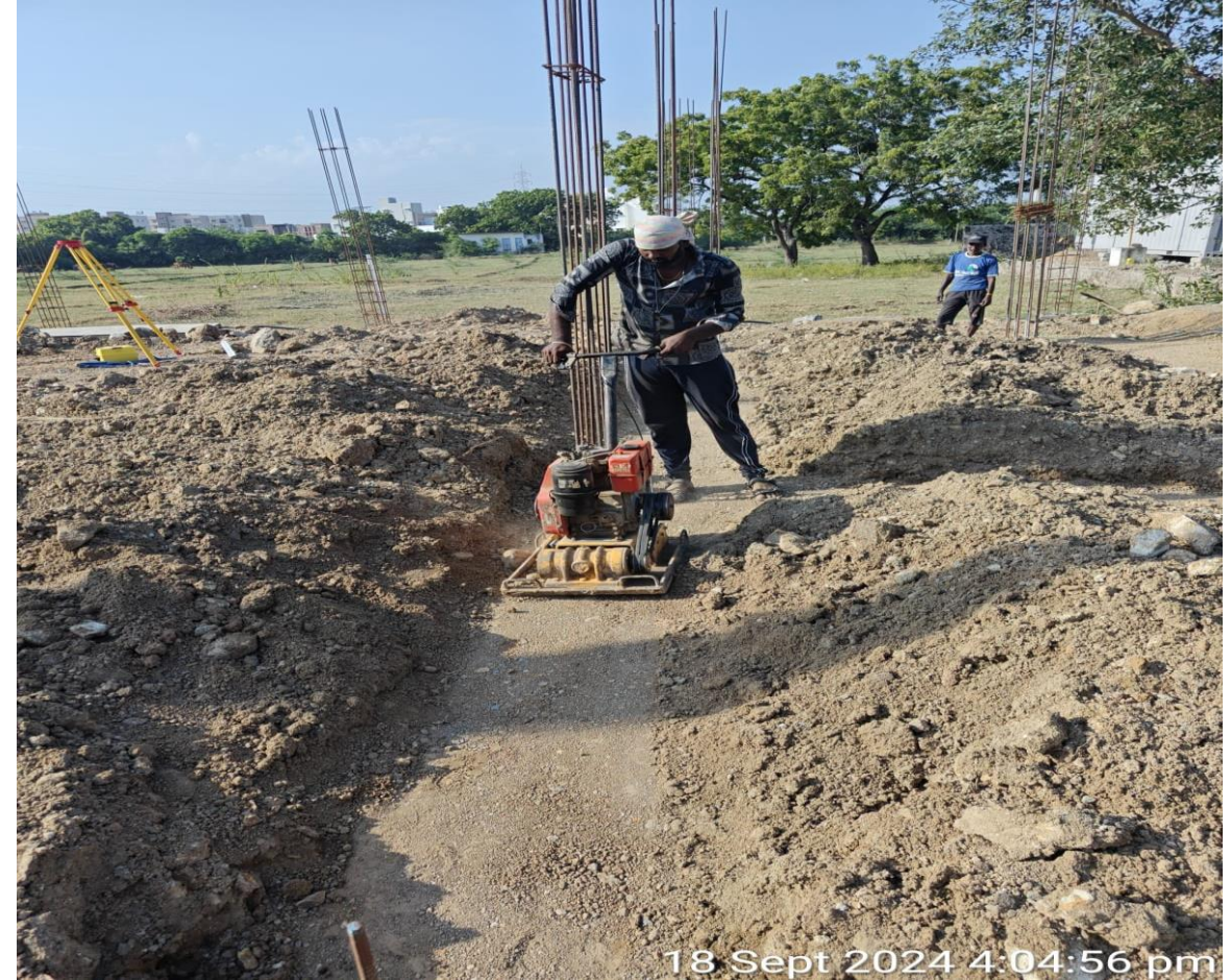
Villa No.16 Plinth beam Bottom soil compaction
