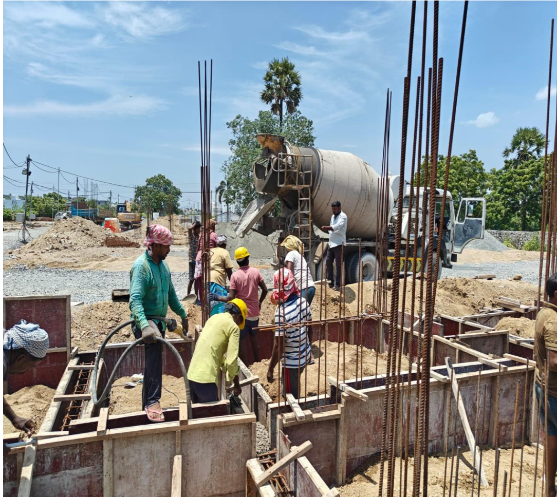
Villa No.20 Plinth Beam Concrete & Deshuttering
