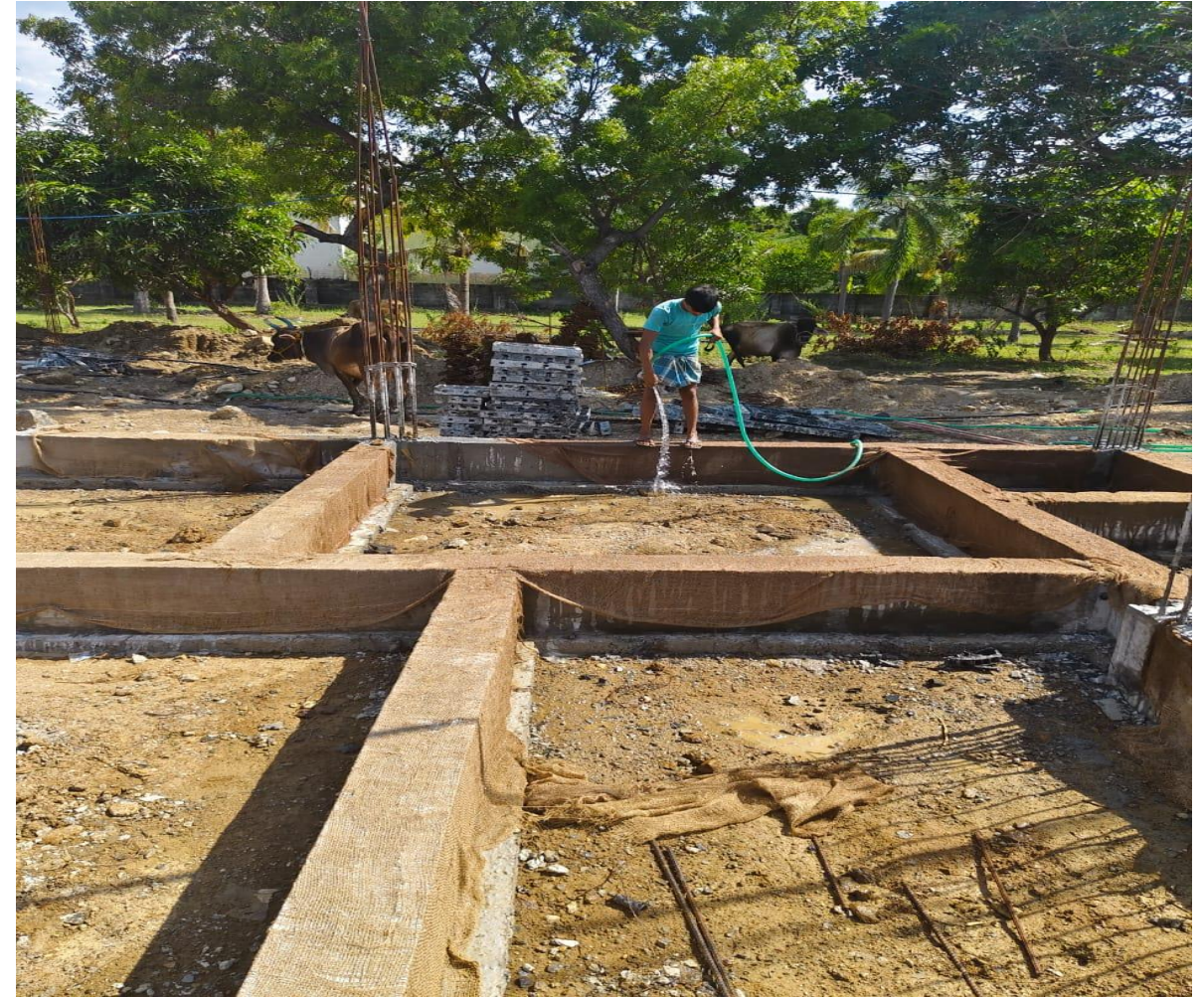
Villa No.06 Plinth beam Concrete
