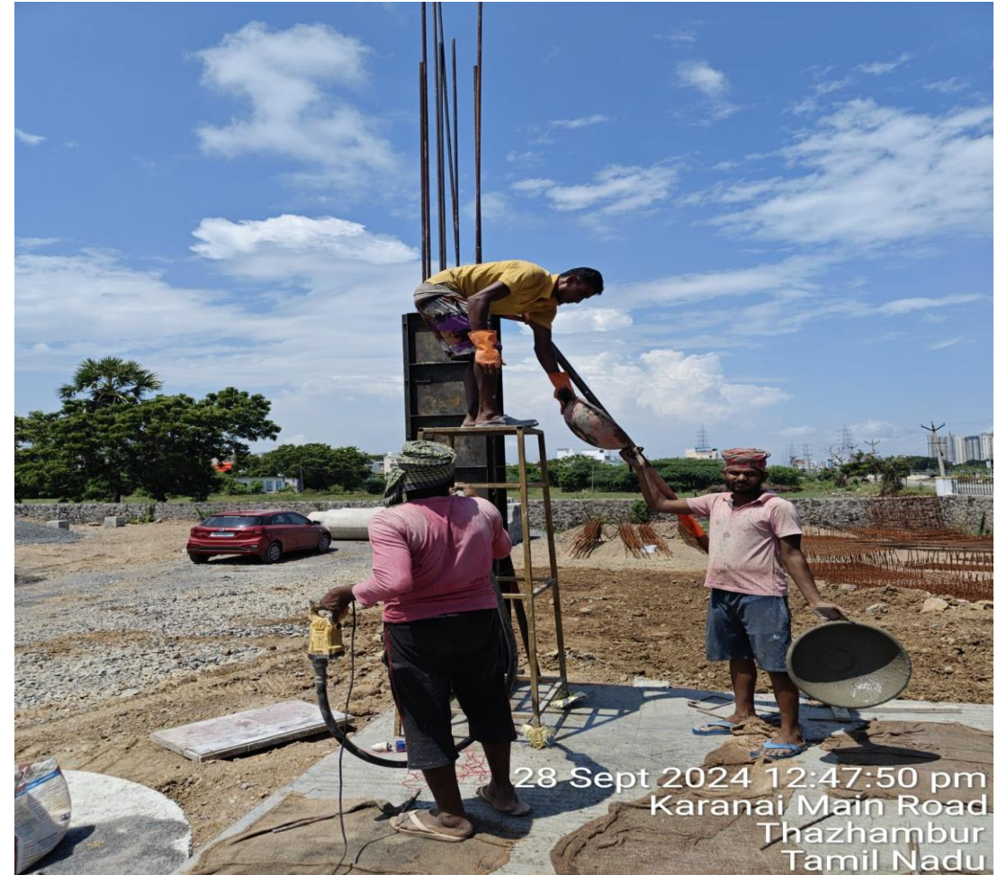
Villa No.20 GF Column shuttering & concrete
