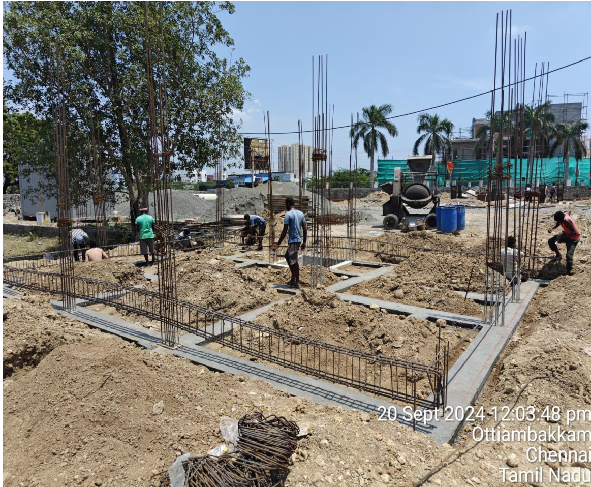
Villa No.16 Plinth Beam Reinforcement steel
