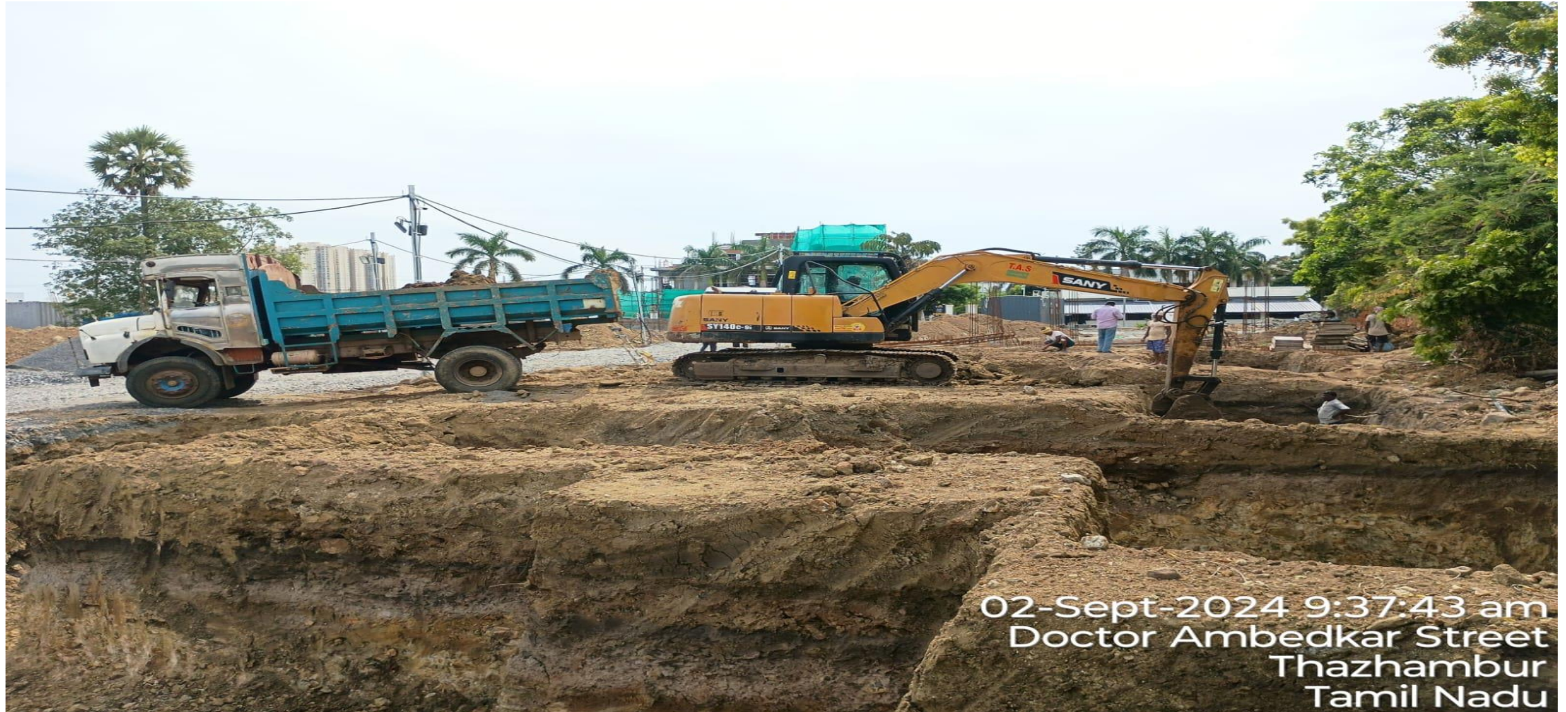
Villa No.09 Footing Earthwork Excavation
