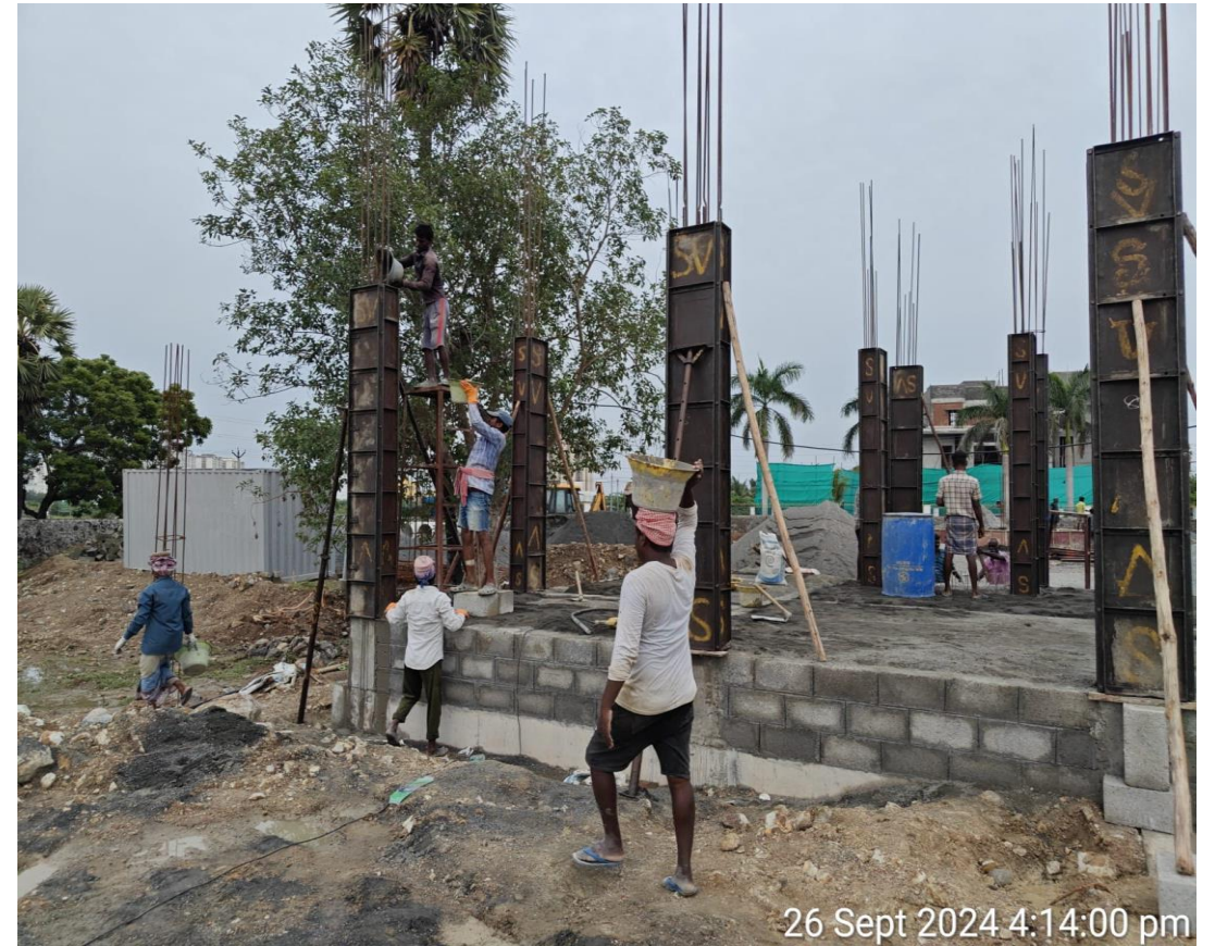
Villa No.16 GF Column Shuttering & Concrete
