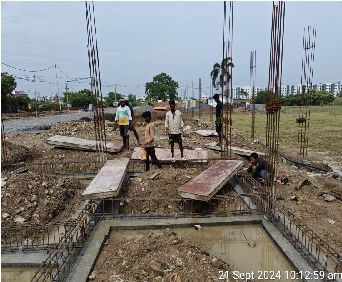
Villa No.16 Plinth Beam Shuttering
