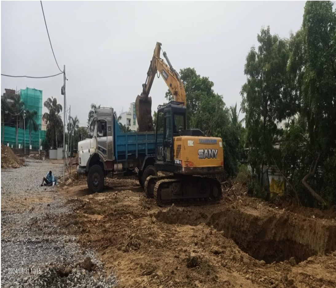
Villa No.10 Earthwork Excavation & Quarry dust filling
