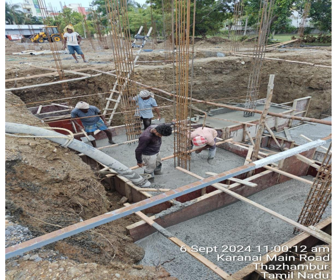
Villa No.08 Footing Reinforcement steel & Concrete
