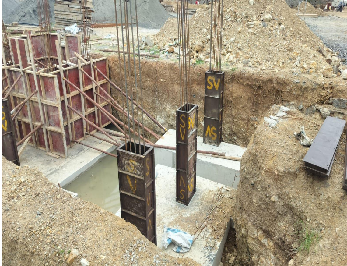
Villa No.16 Pedestal column Shuttering & Concrete
