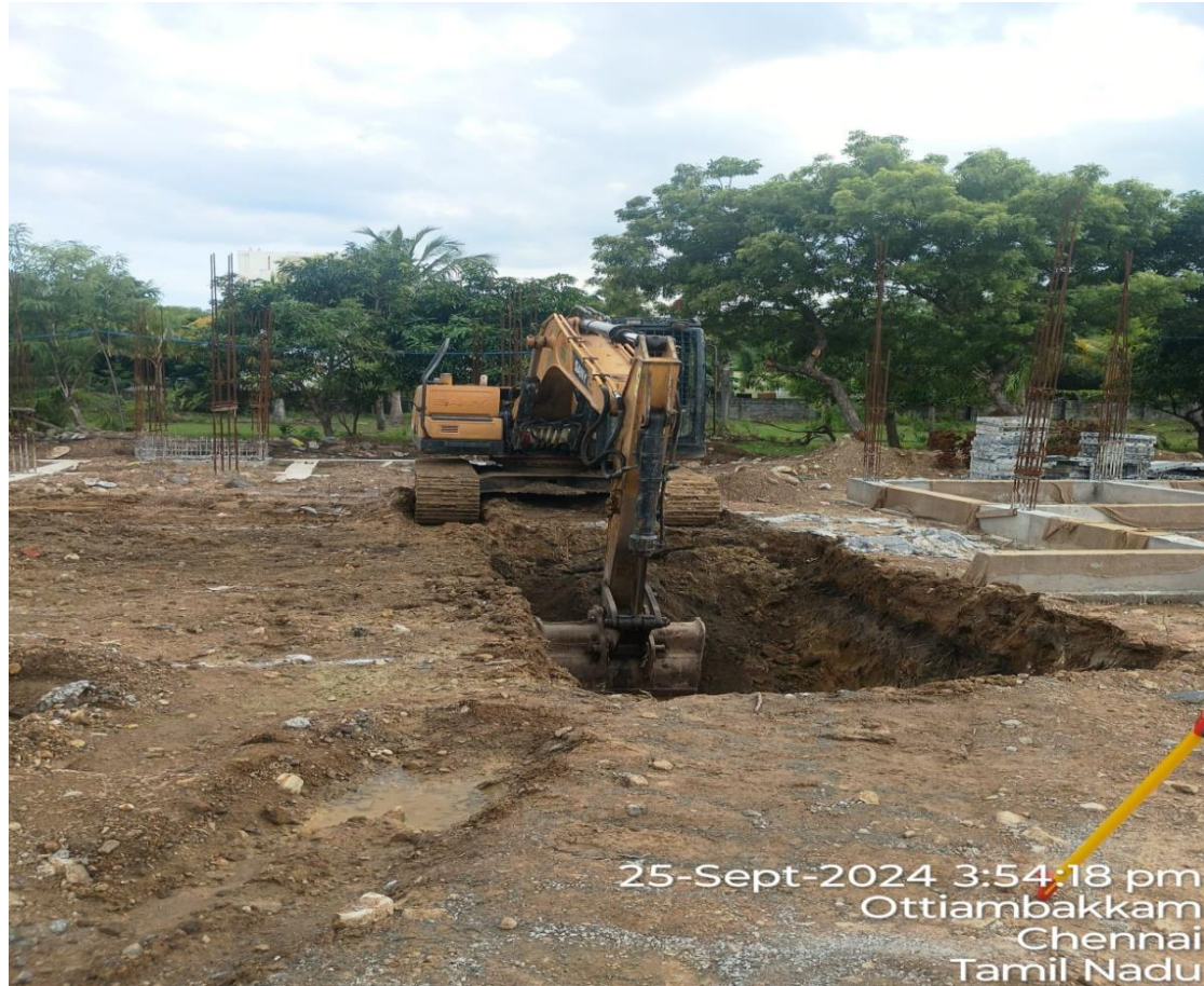
Villa No.05 Footing Earthwork Excavation
