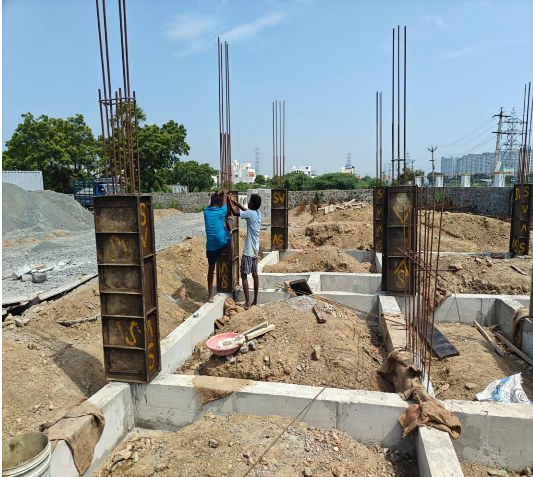
Villa No.20 Basement column Shuttering & concrete Block work
