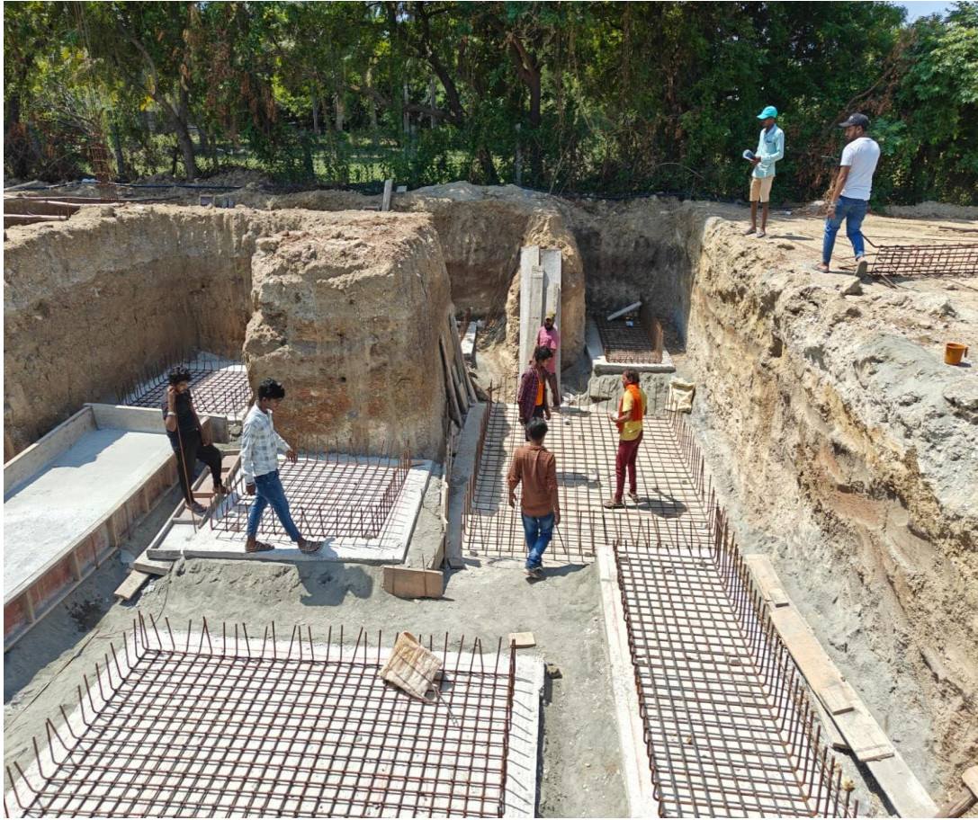
Villa No.11 Footing Reinforcement Steel
