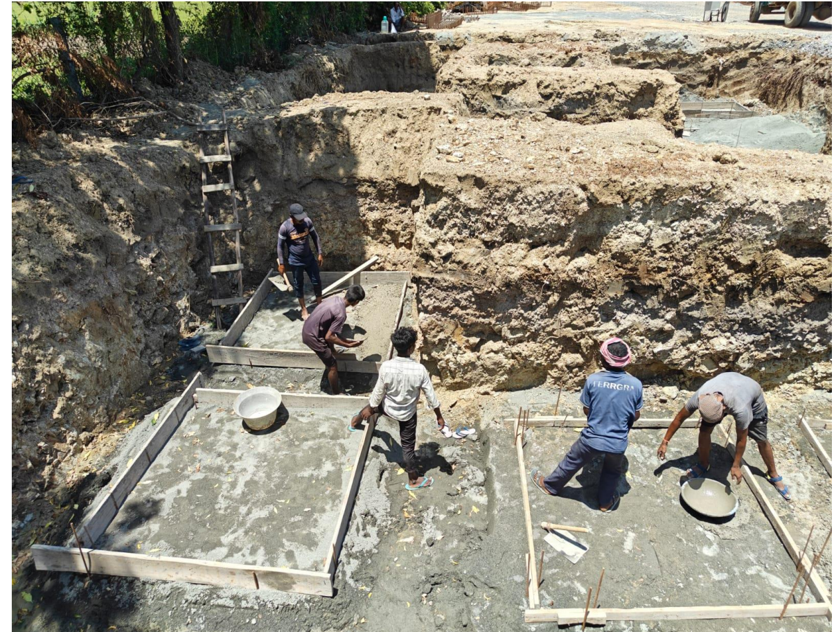
Villa No.10 Earthwork Excavation & Quarry dust filling
