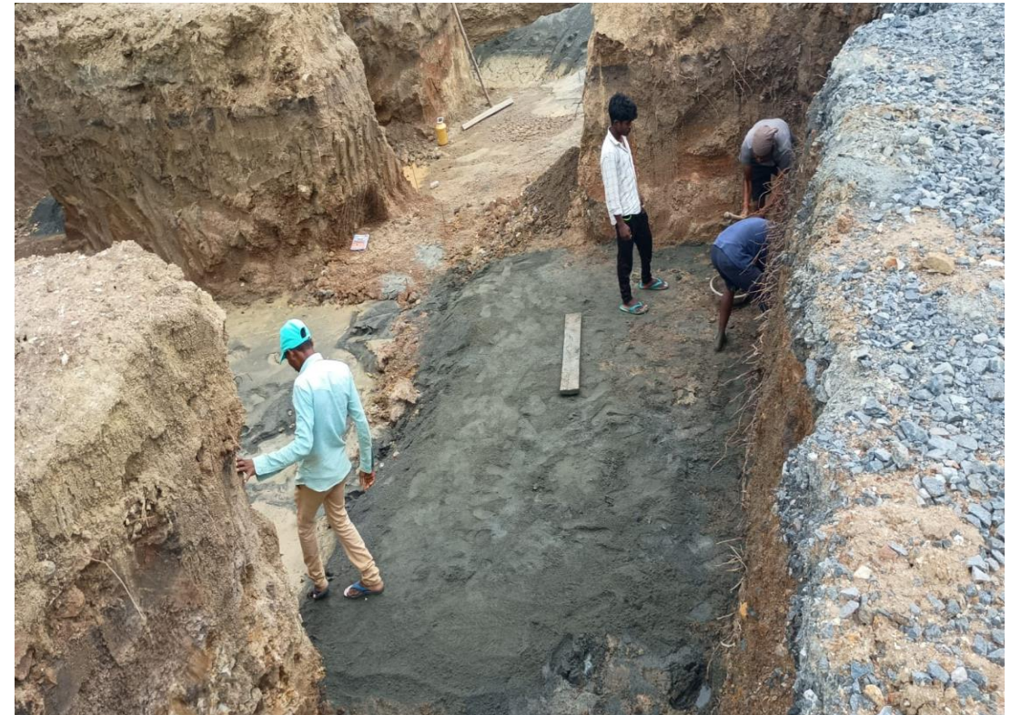
Villa No.11 Footing Earthwork excavation & Quarry dust filling work
