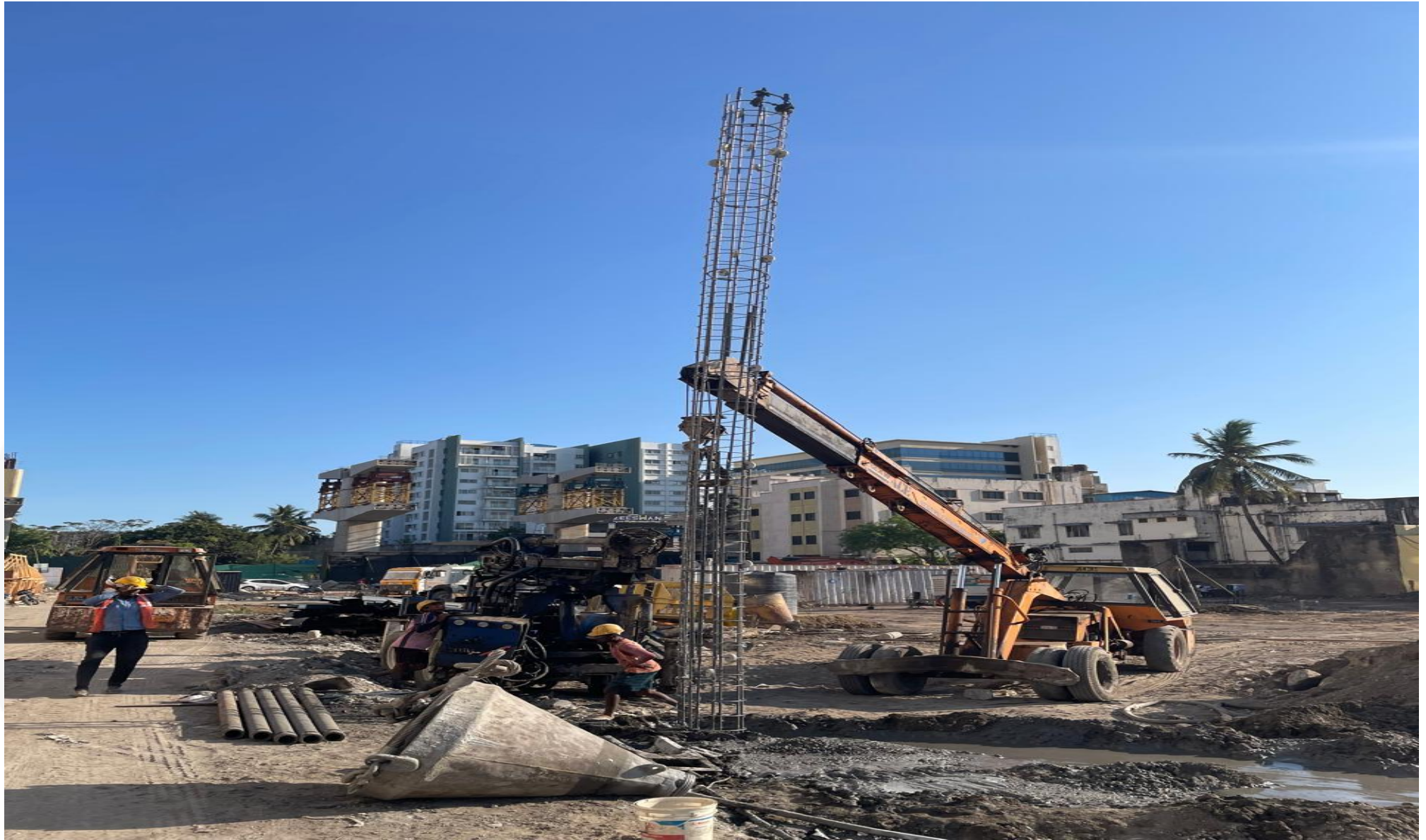
Contiguous Pile Reinforcement Work In Progress
