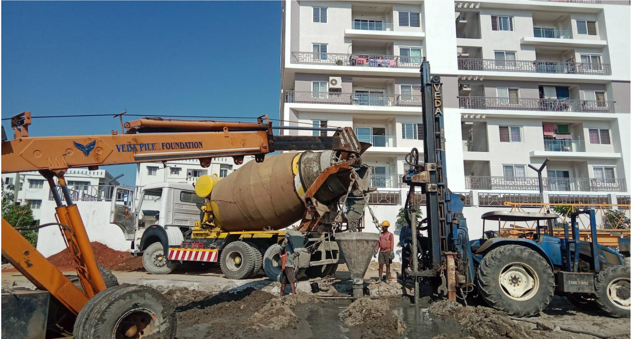
Contiguous Pile Concreting Work In Progress
