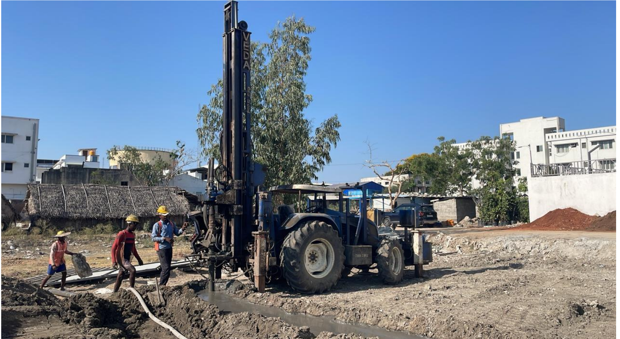
Contiguous Pile Boring Work In Progress
