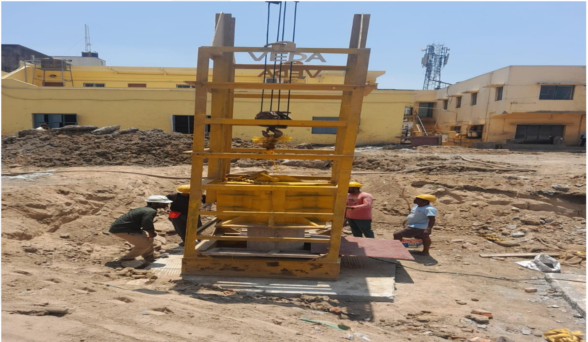
Pile Dynamic Load Test Completed
