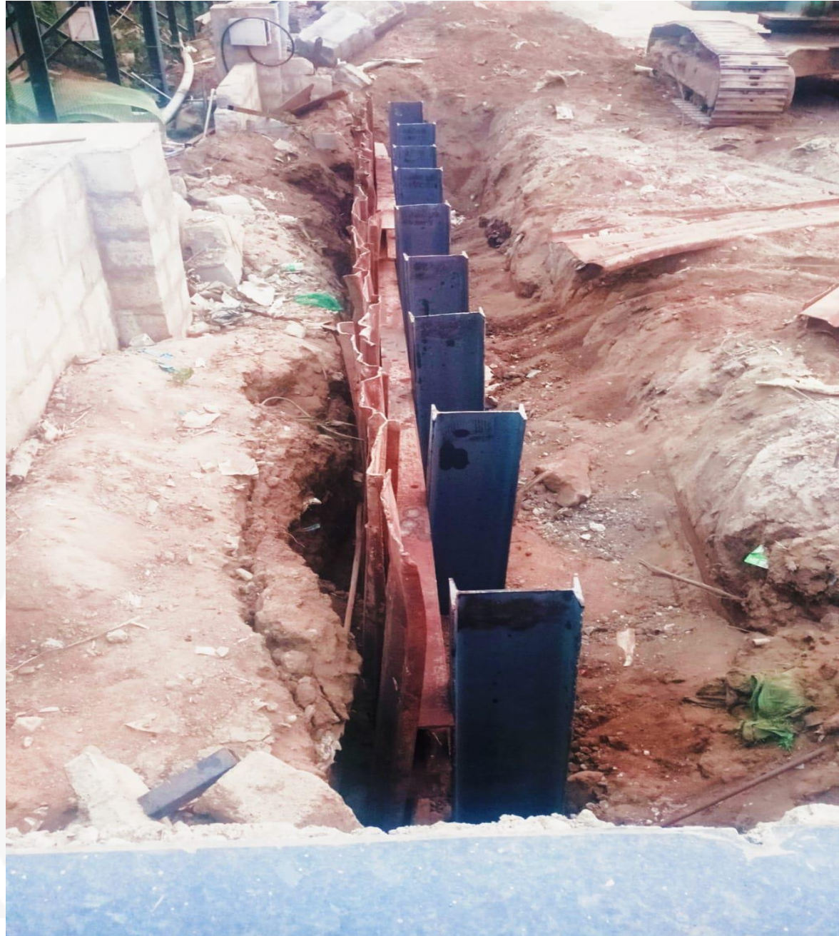
Shoring Work In Progress
