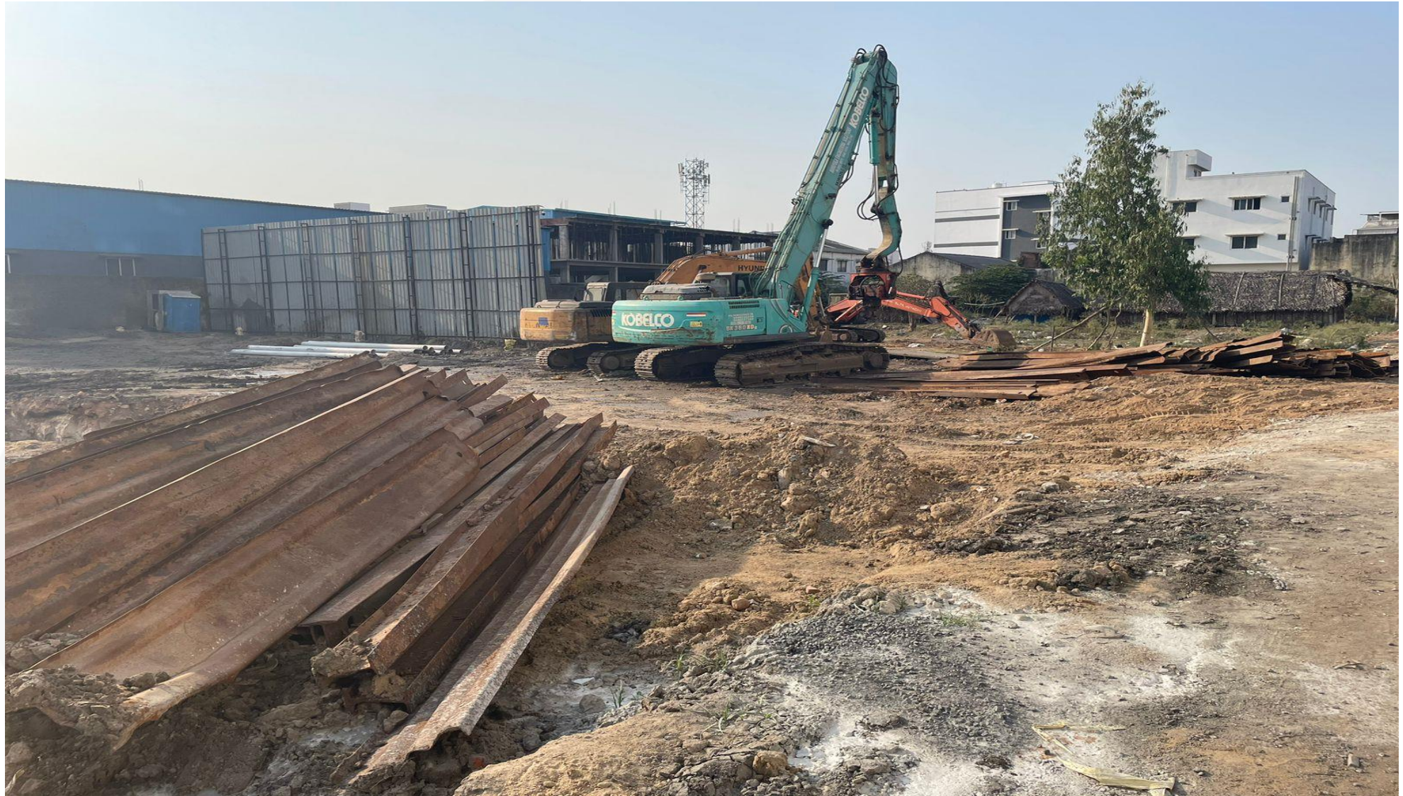
Shoring Work Commenced
