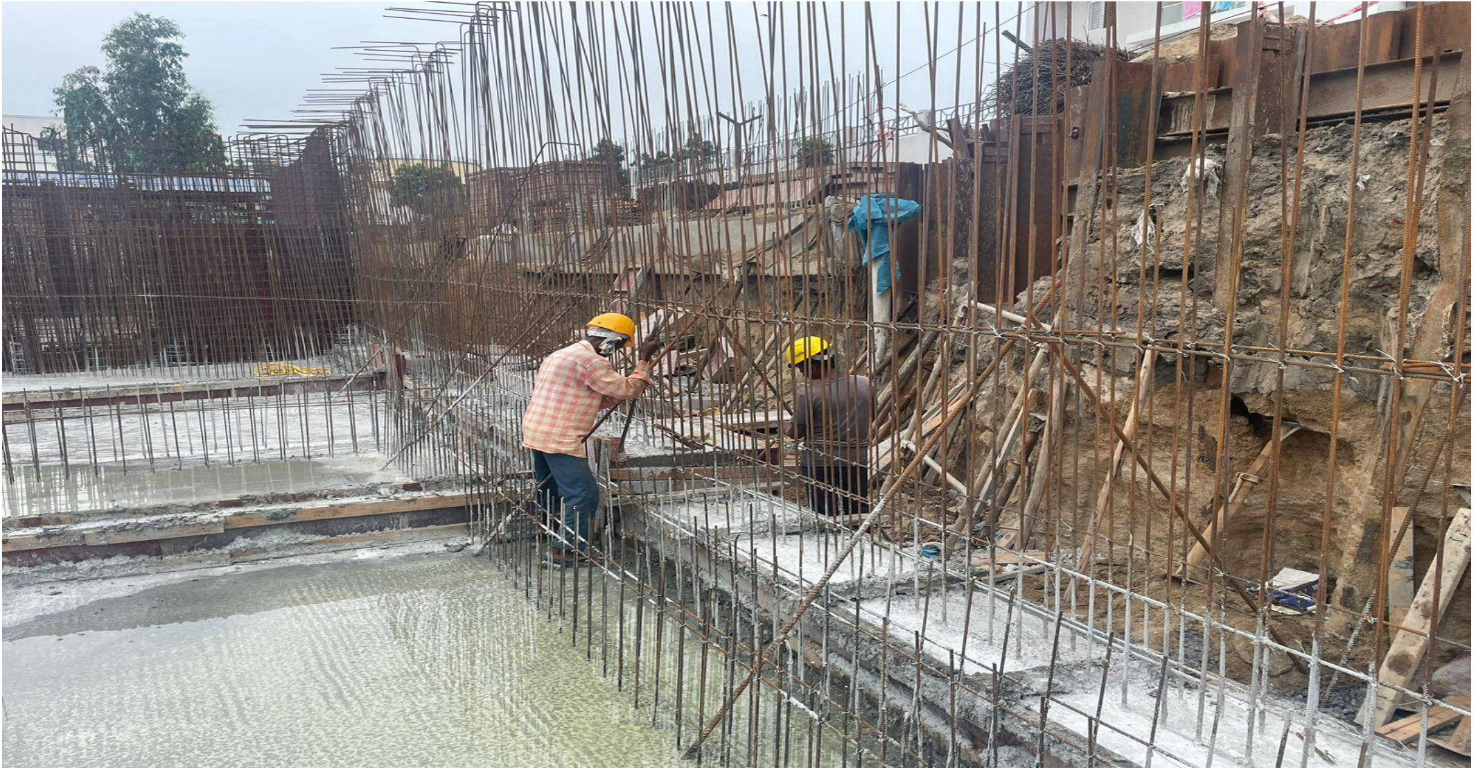
Basement P-01 Raft de-shuttering work completed.
