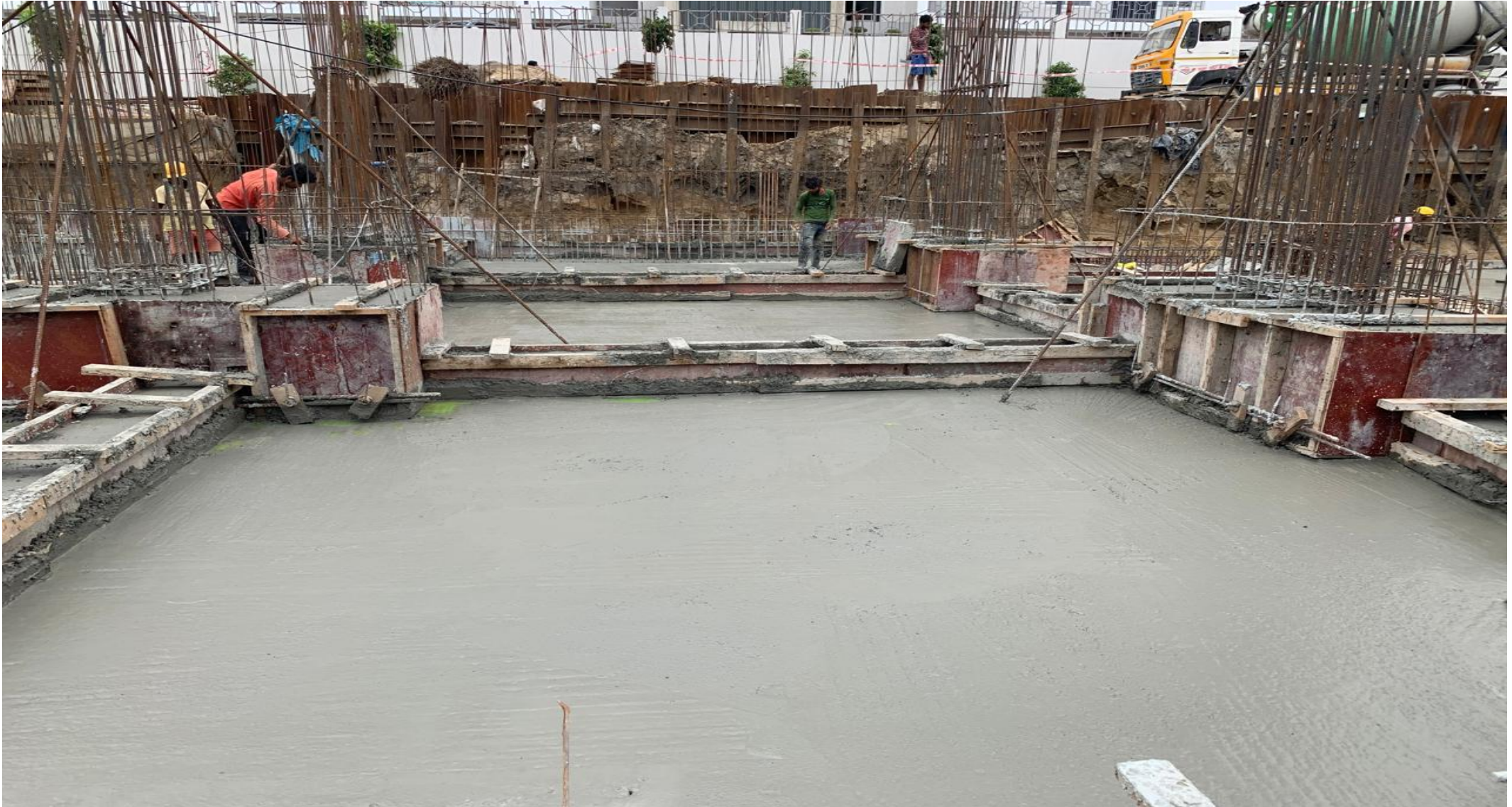
Basement P-01 Raft Concrete work completed.
