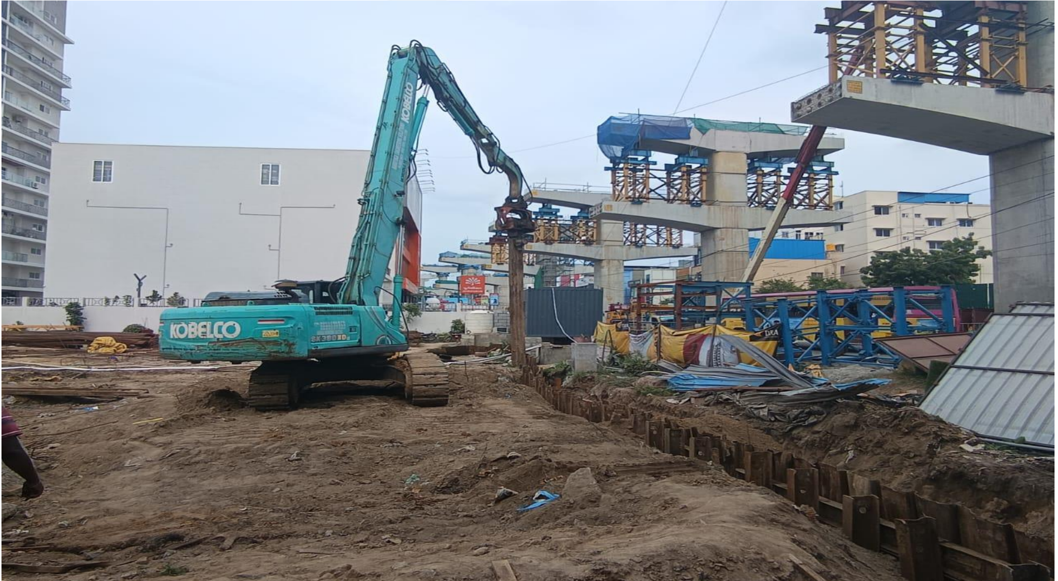
Sheet pile shoring work completed.
