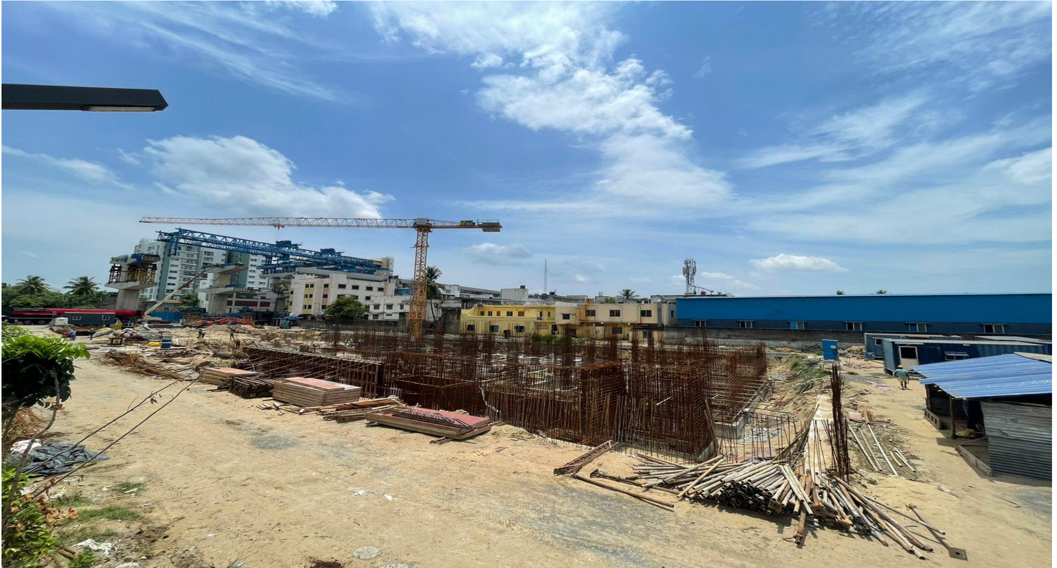
North East corner view.
