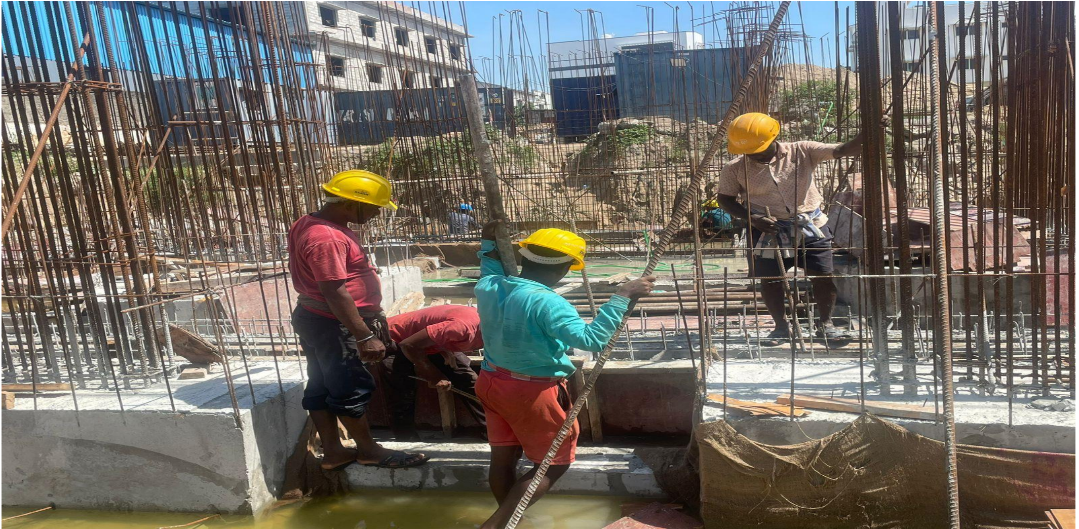
Basement P-01 UG Sump raft slab de-shuttering work completed.
