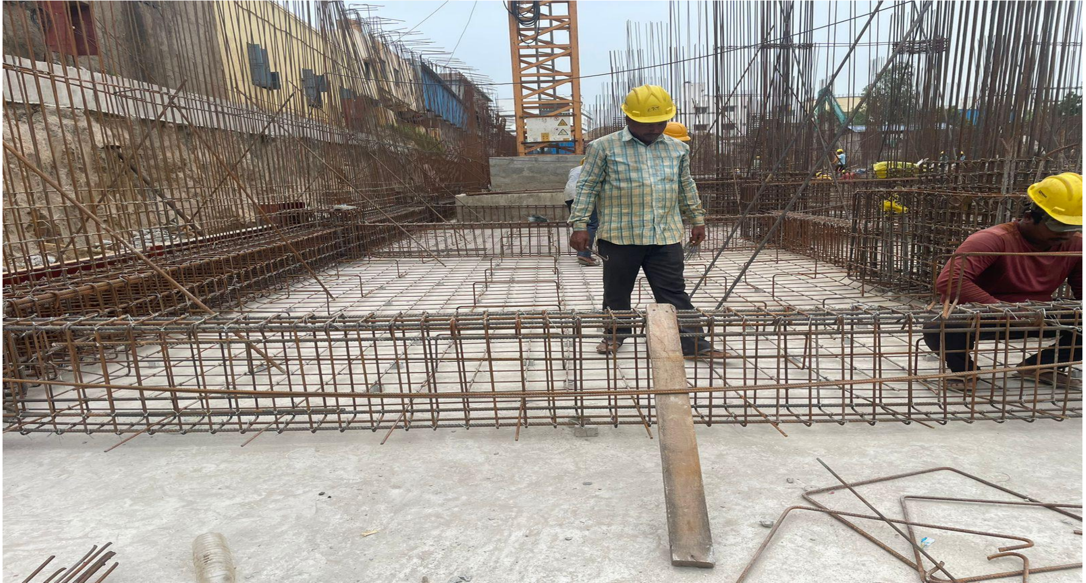
Pour-02 Raft, pile cap & beam reinforcement work in progress.
