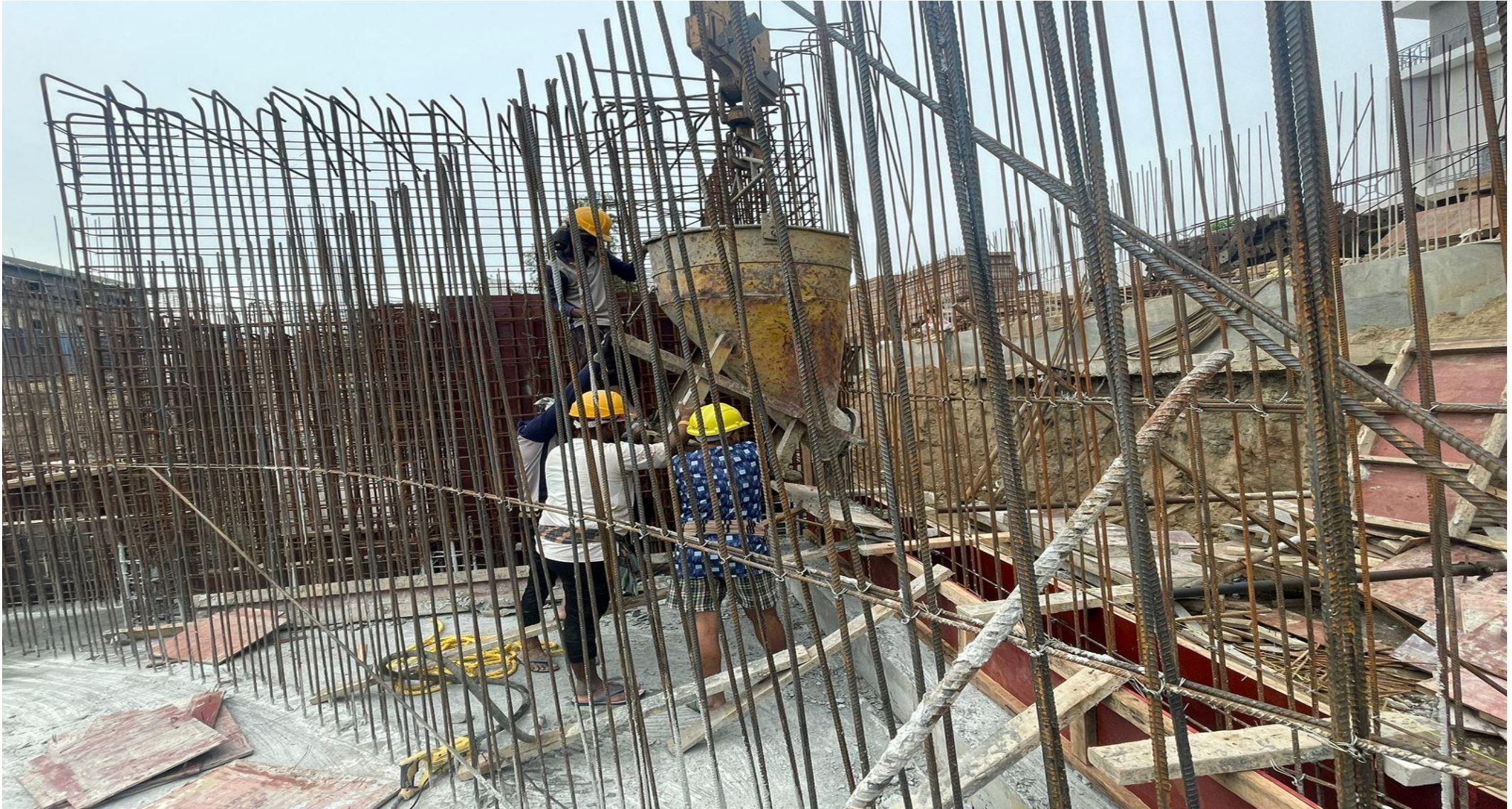
East side retaining wall starter Concrete work completed.
