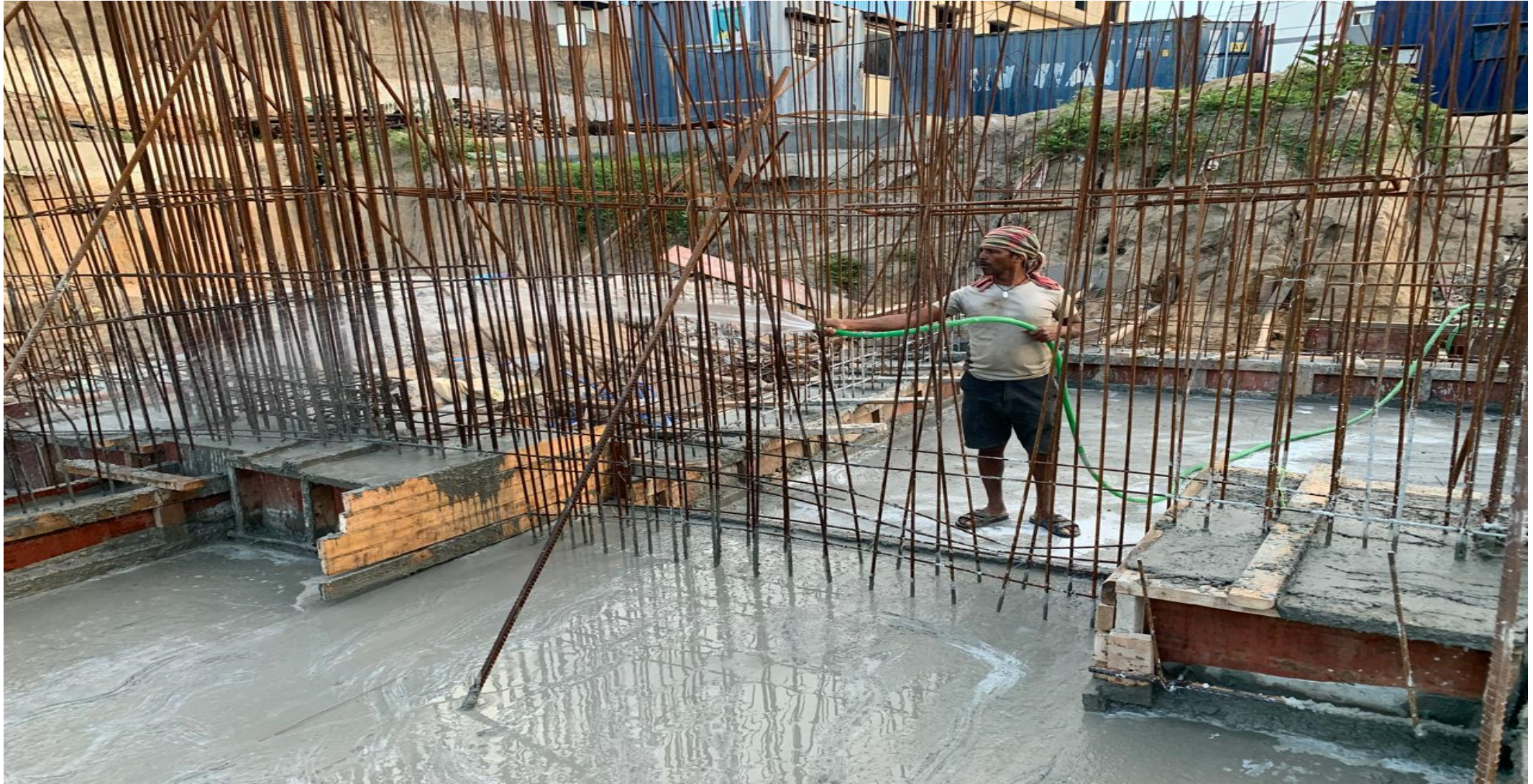
Basement P-01 UG Sump raft slab curing work in progress.
