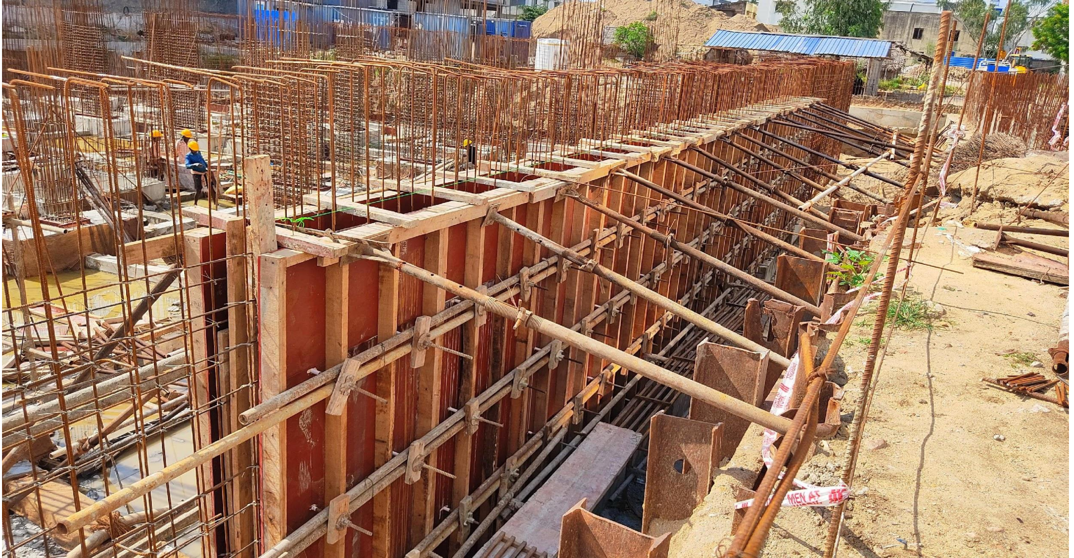
East side retaining wall shuttering work in progress.
