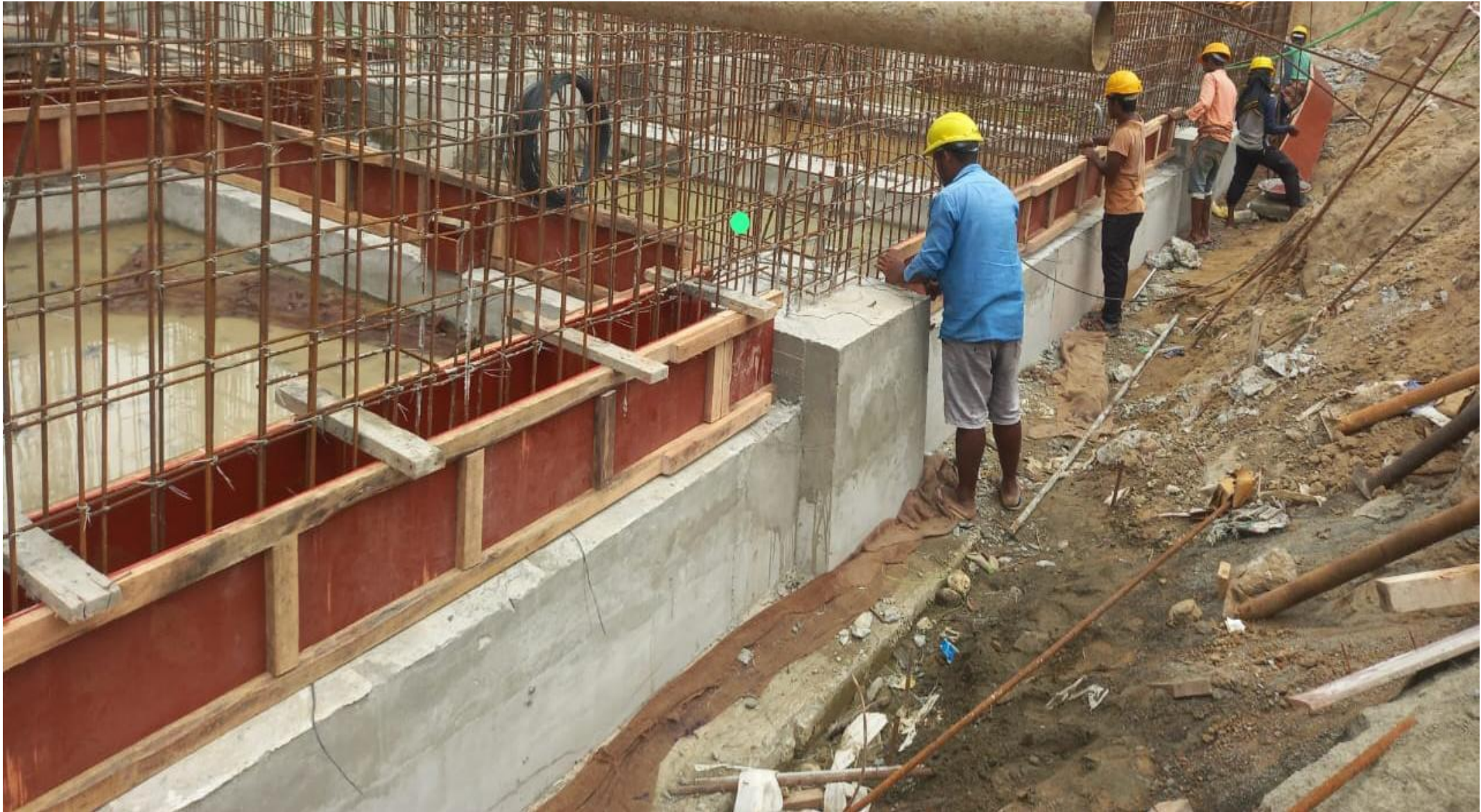
East side retaining wall starter shuttering work completed.
