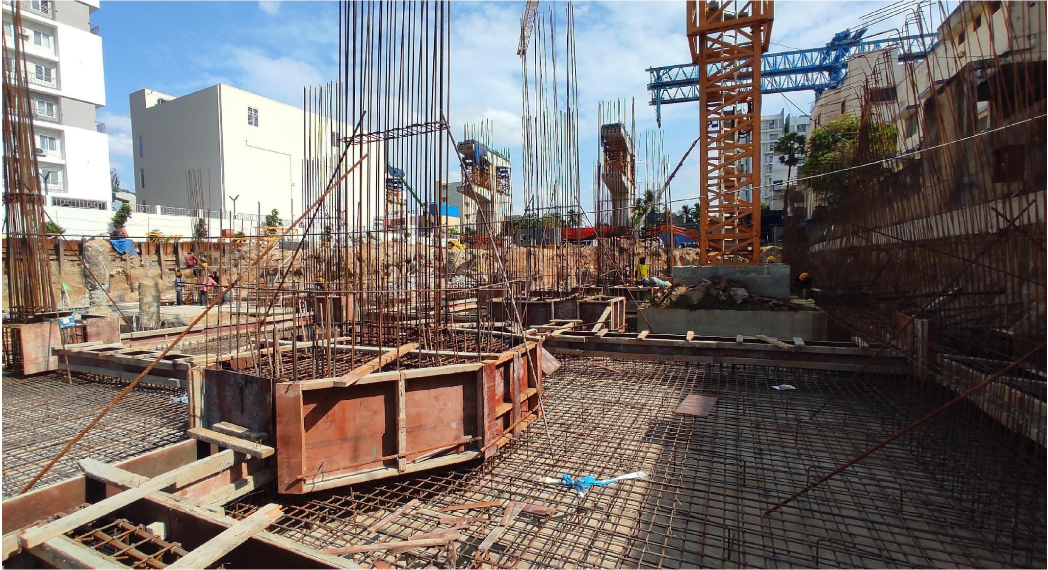
Pour-02 area shuttering work in progress.
