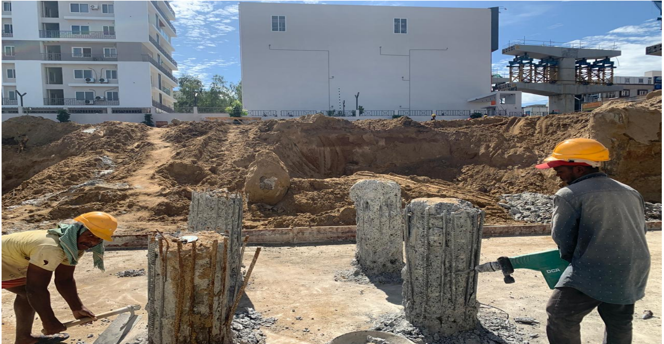
Pour -02 & 03 area PCC completed, pile chipping work in progress.
