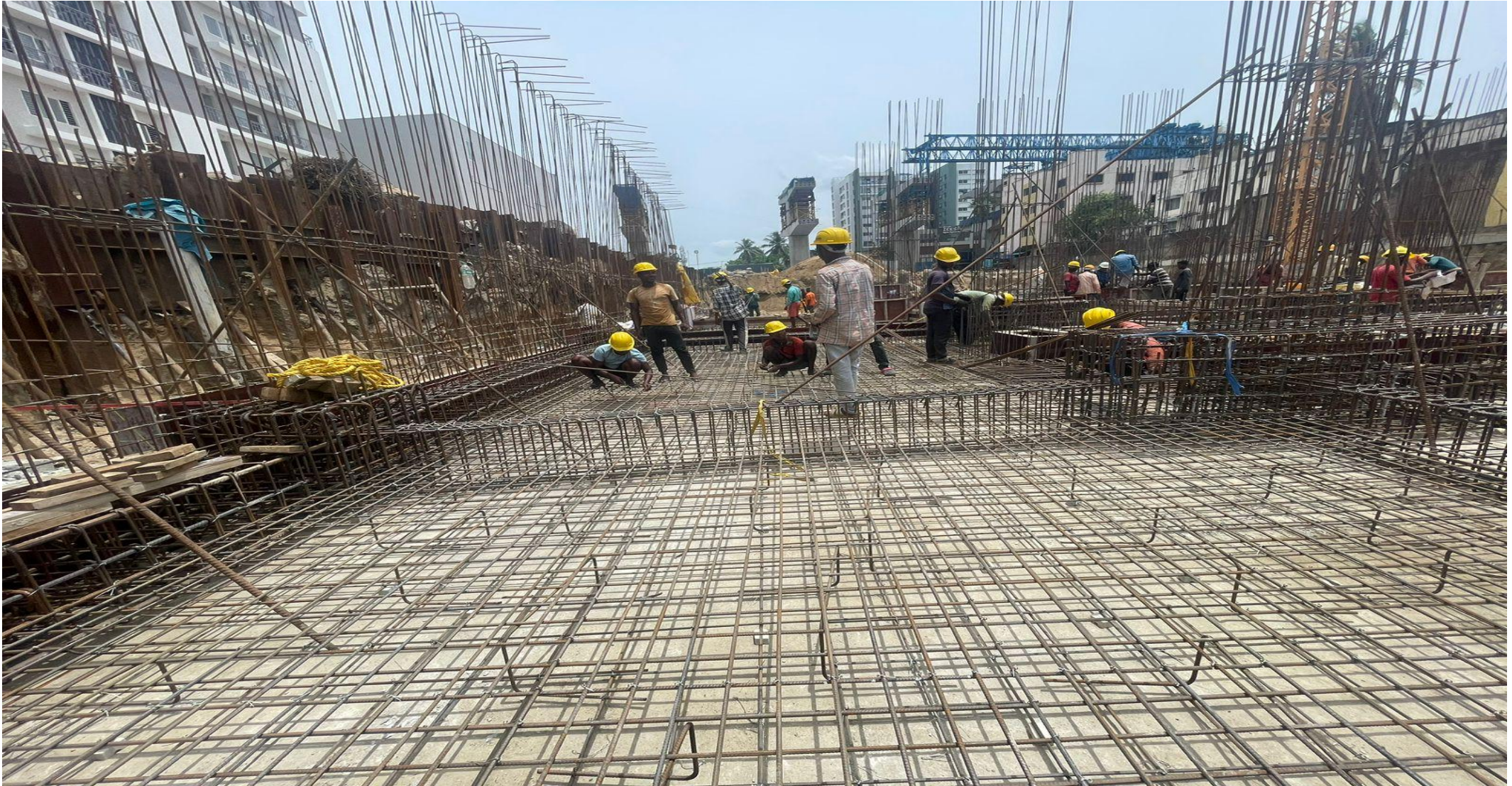
Basement Pour 1 raft slab reinforcement work in progress.
