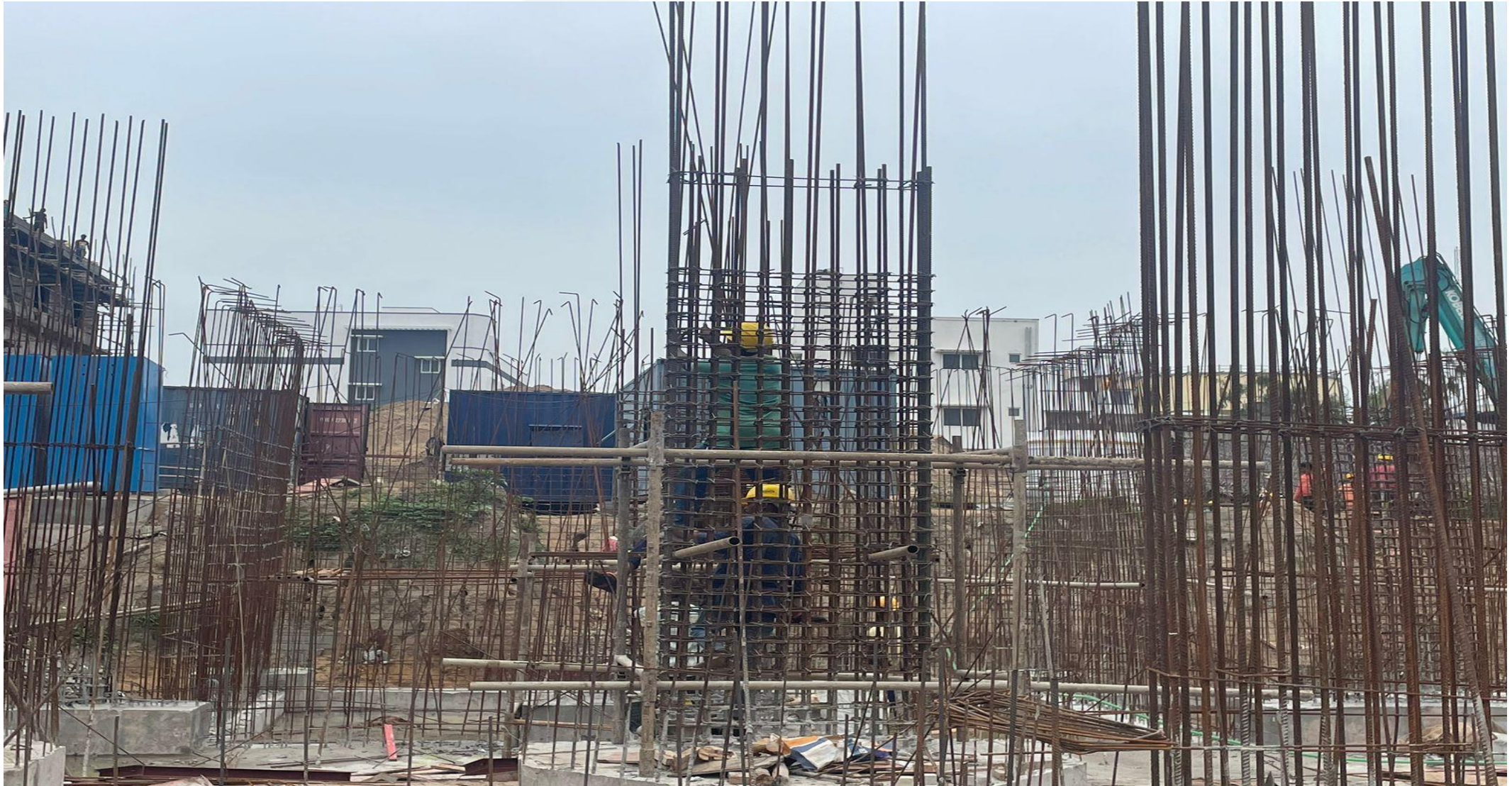
Pour-01 area column reinforcement work in progress.
