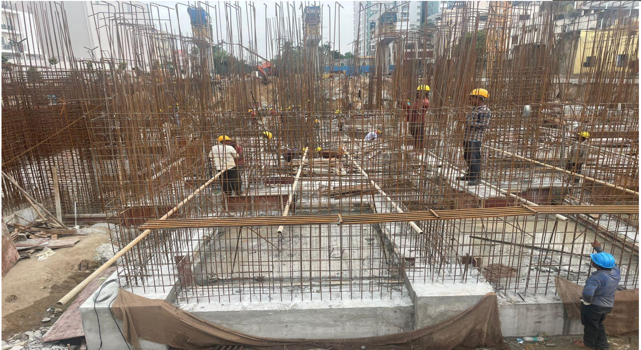
Basement P-01 UG Sump around area wall reinforcement work in progress.
