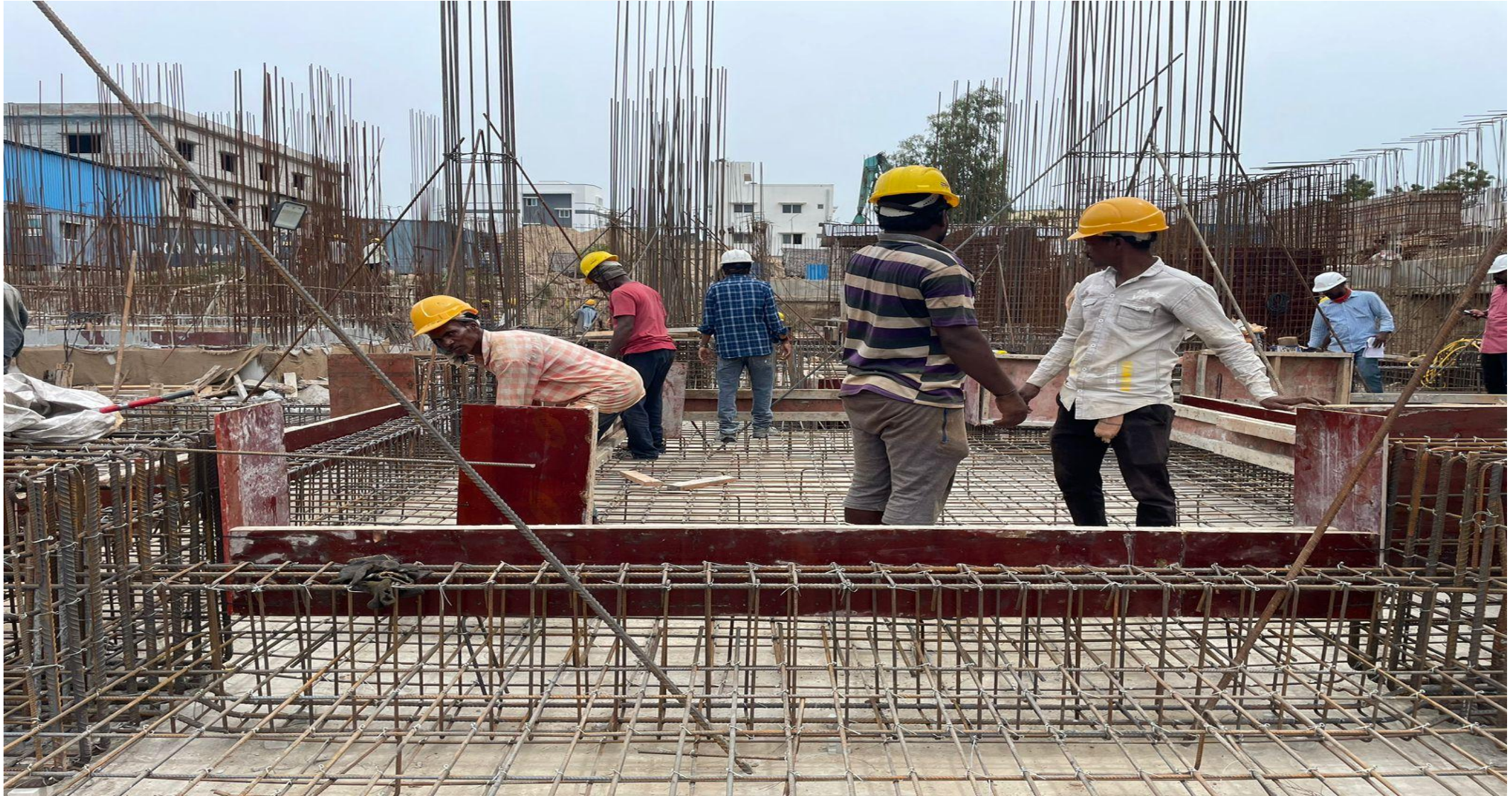
Basement P-01 Raft Pile cap & beam shuttering work in progress.
