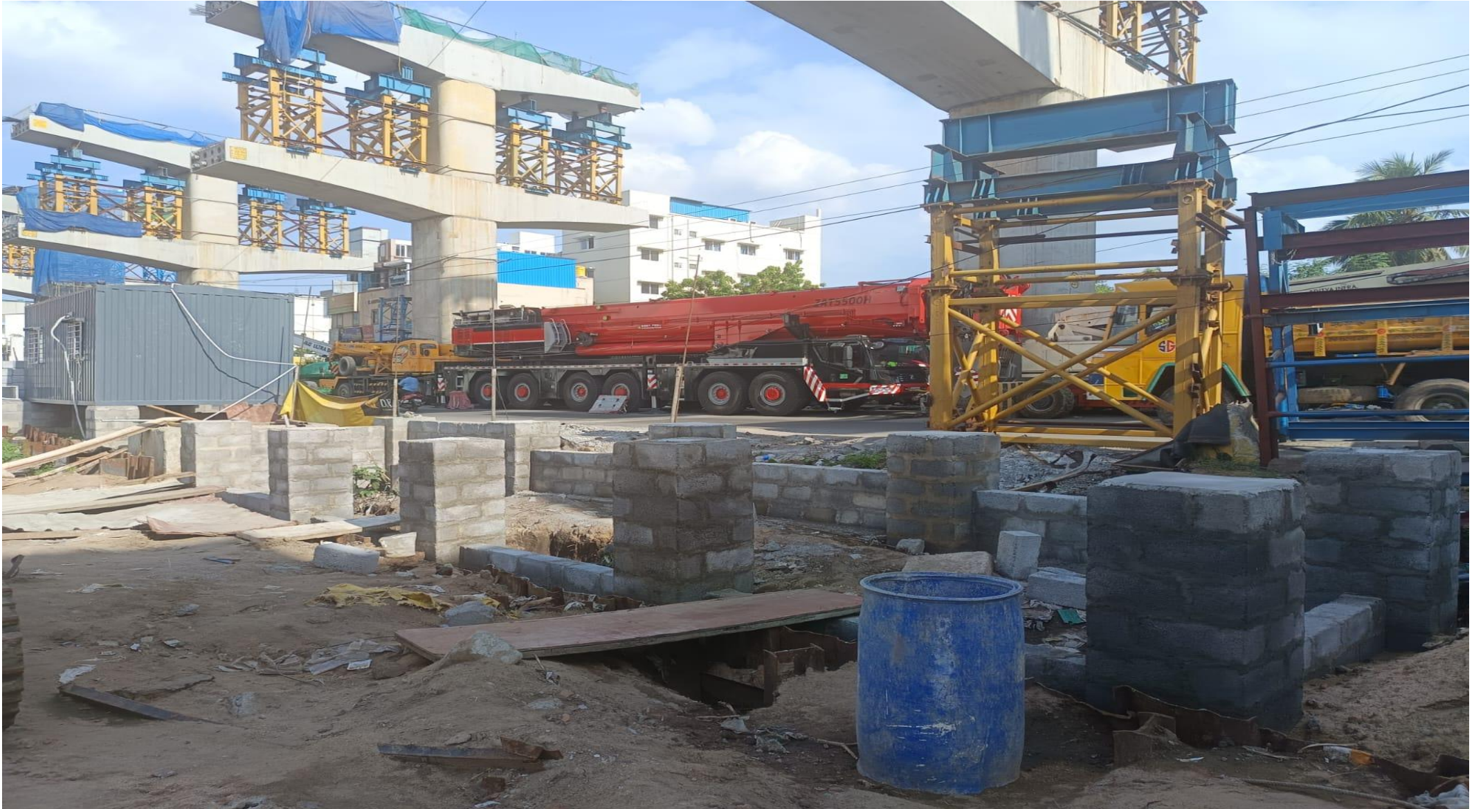
Sales office, foundation work completed.
