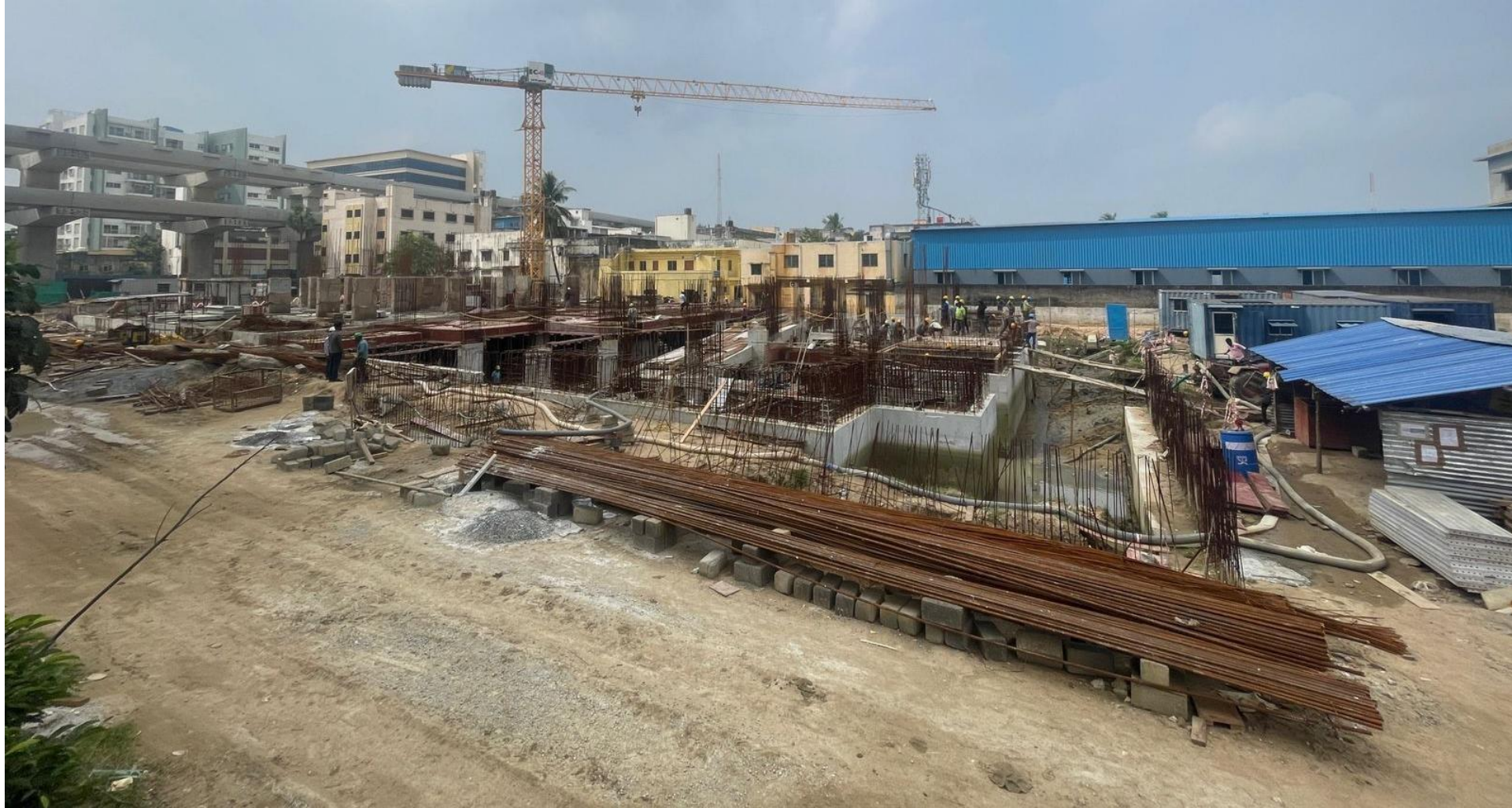
North east corner view.
