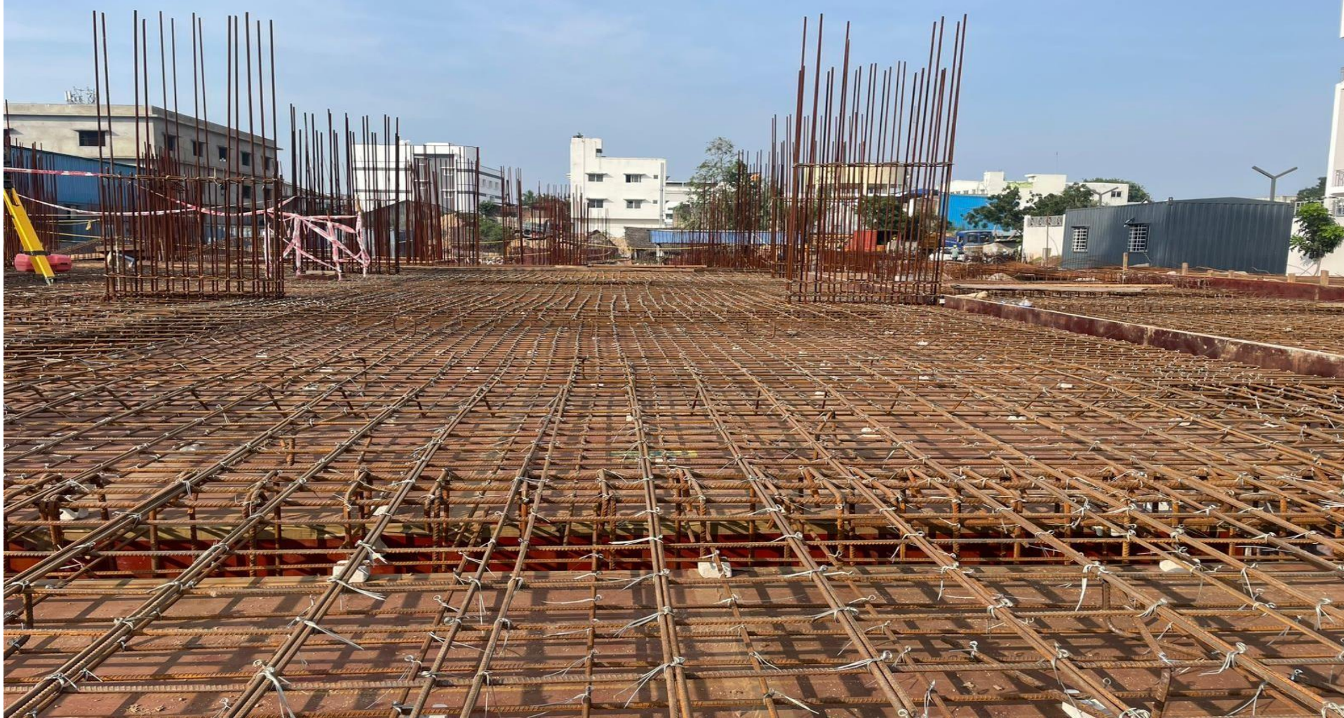
Pour -1 basement roof slab reinforcement work completed.
