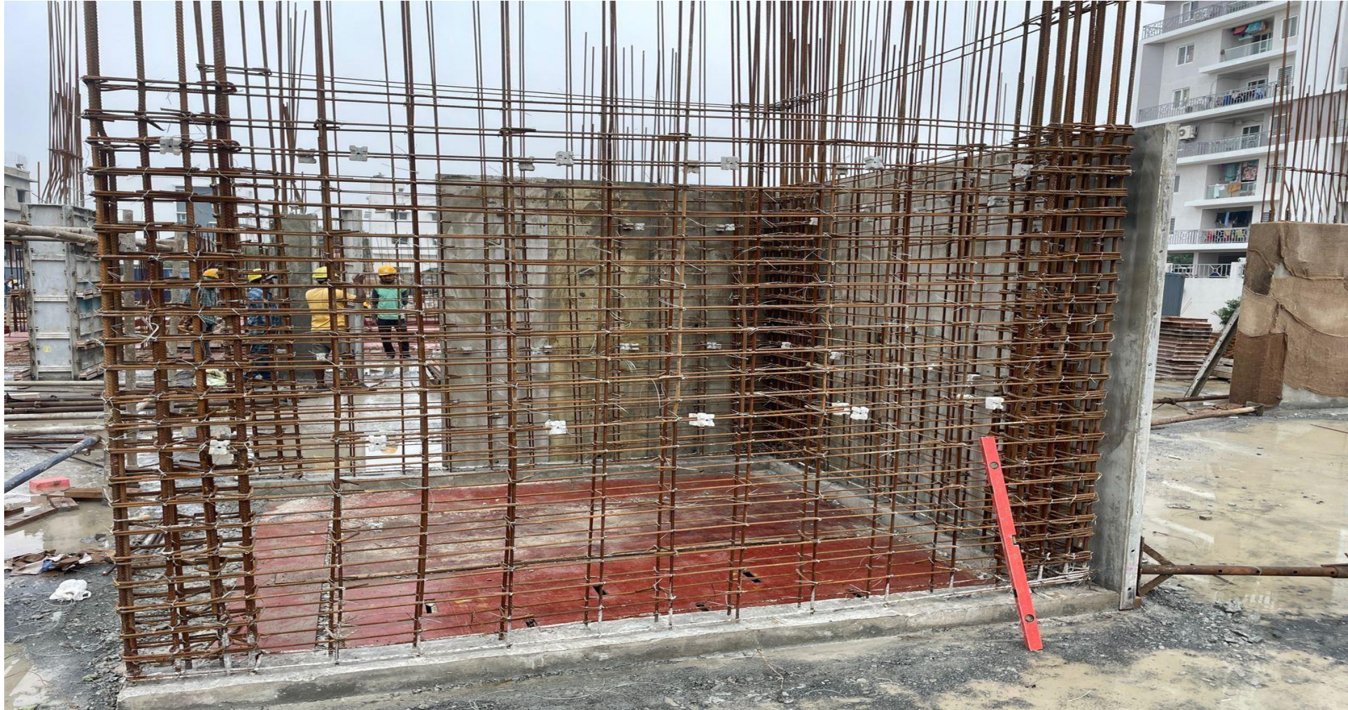
Pour-1 stilt floor lift wall reinforcement work completed.
