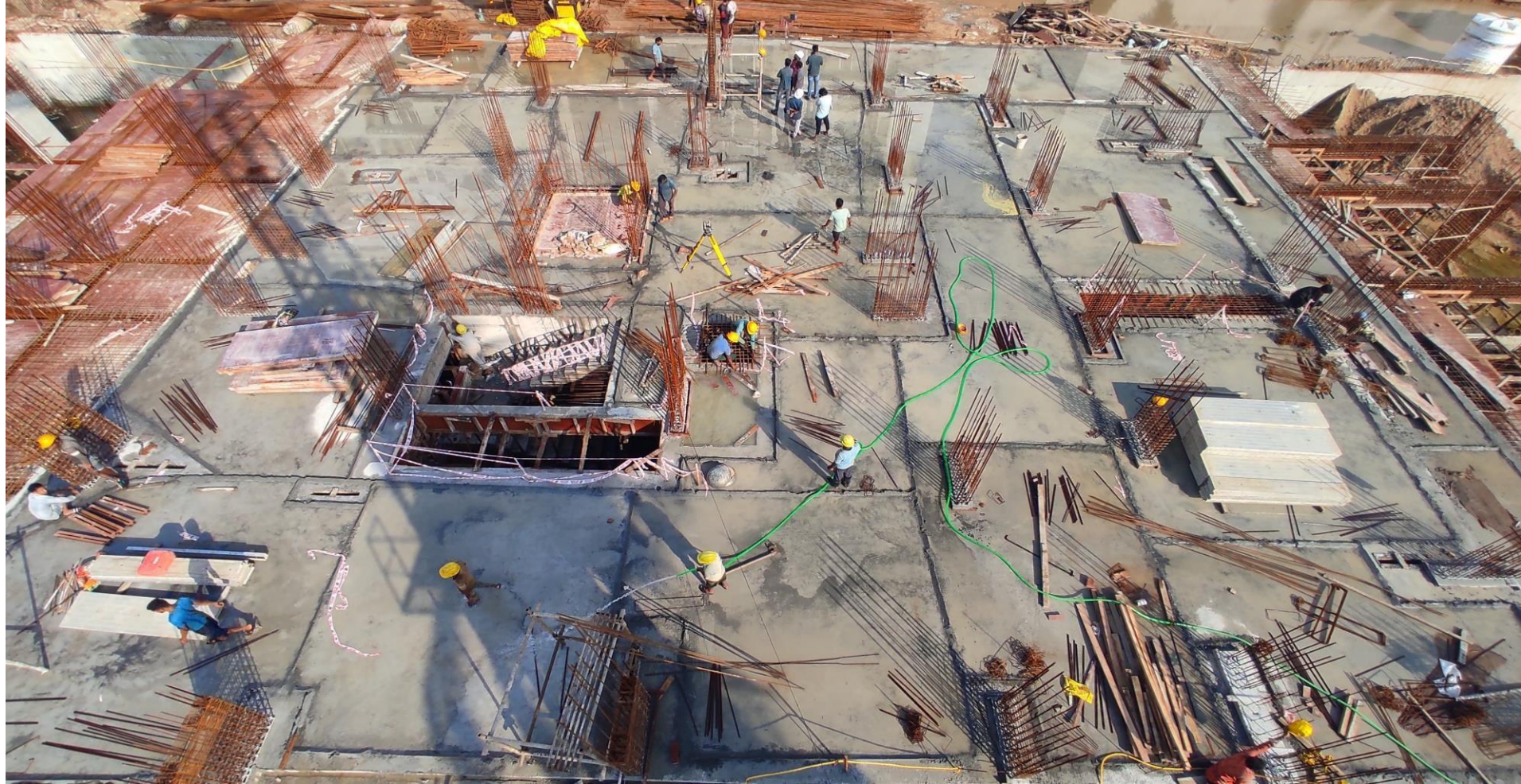
Basement roof slab curing work in progress.
