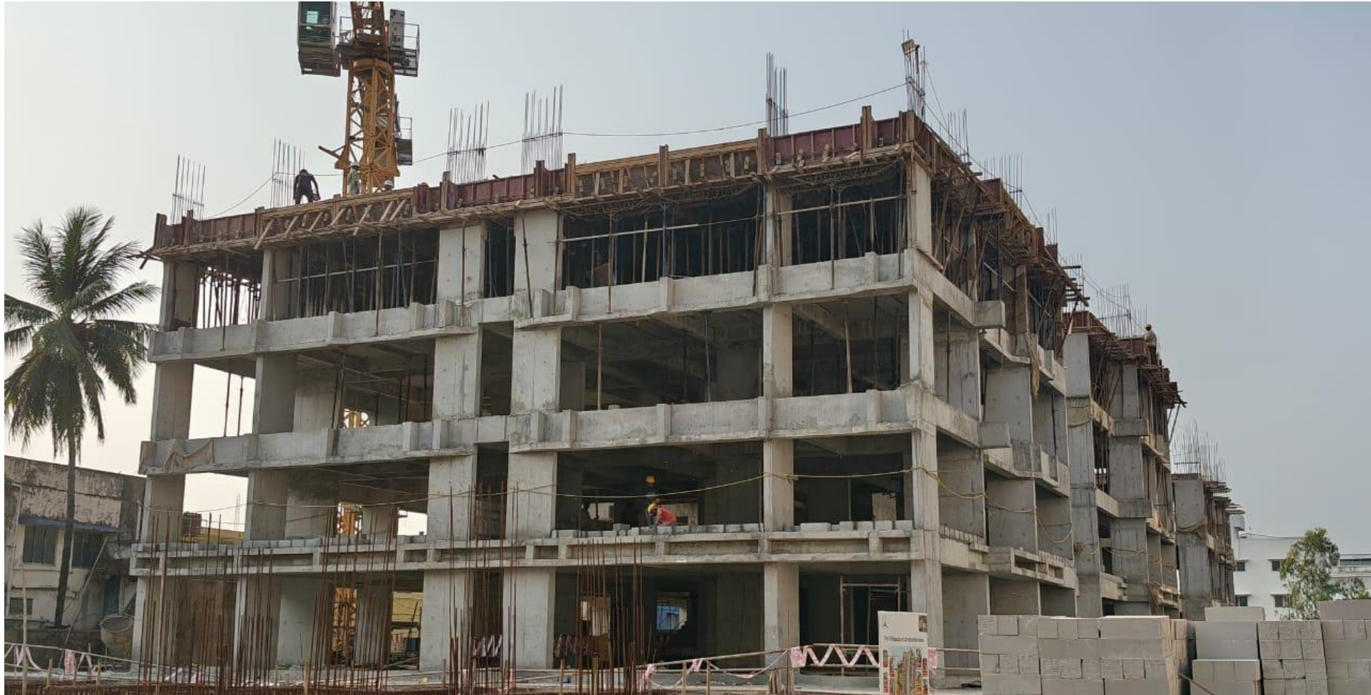
Pour 1 – 3 rd Floor roof outer shuttering work completed.
