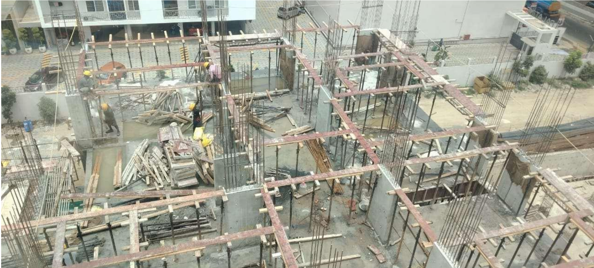
Pour 1 – 4 th Floor roof slab shuttering work in progress.
