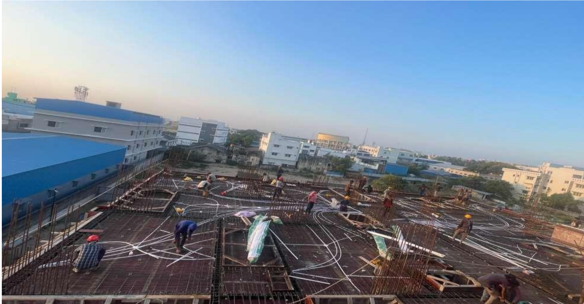
Pour 2 – 2 nd Floor roof electrical conduit laying work completed.
