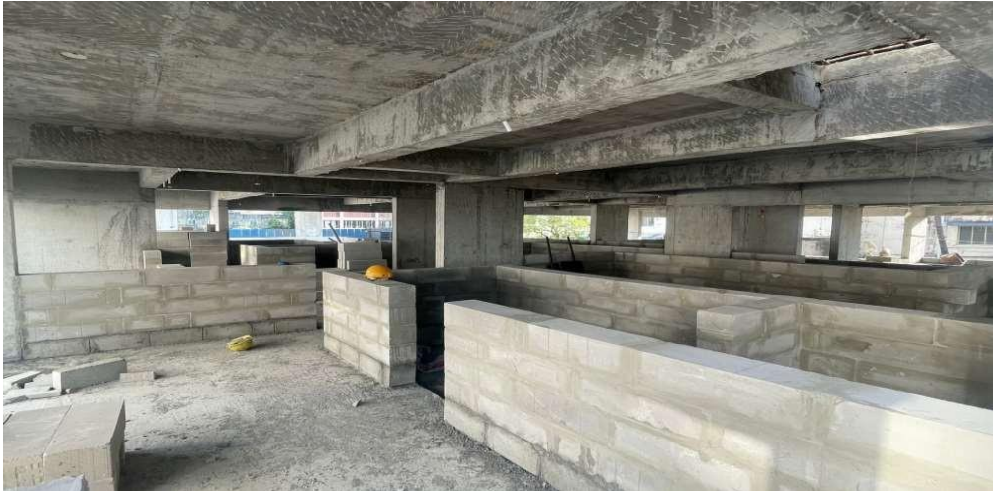
Pour 1 – 1 st Floor block work in progress.
