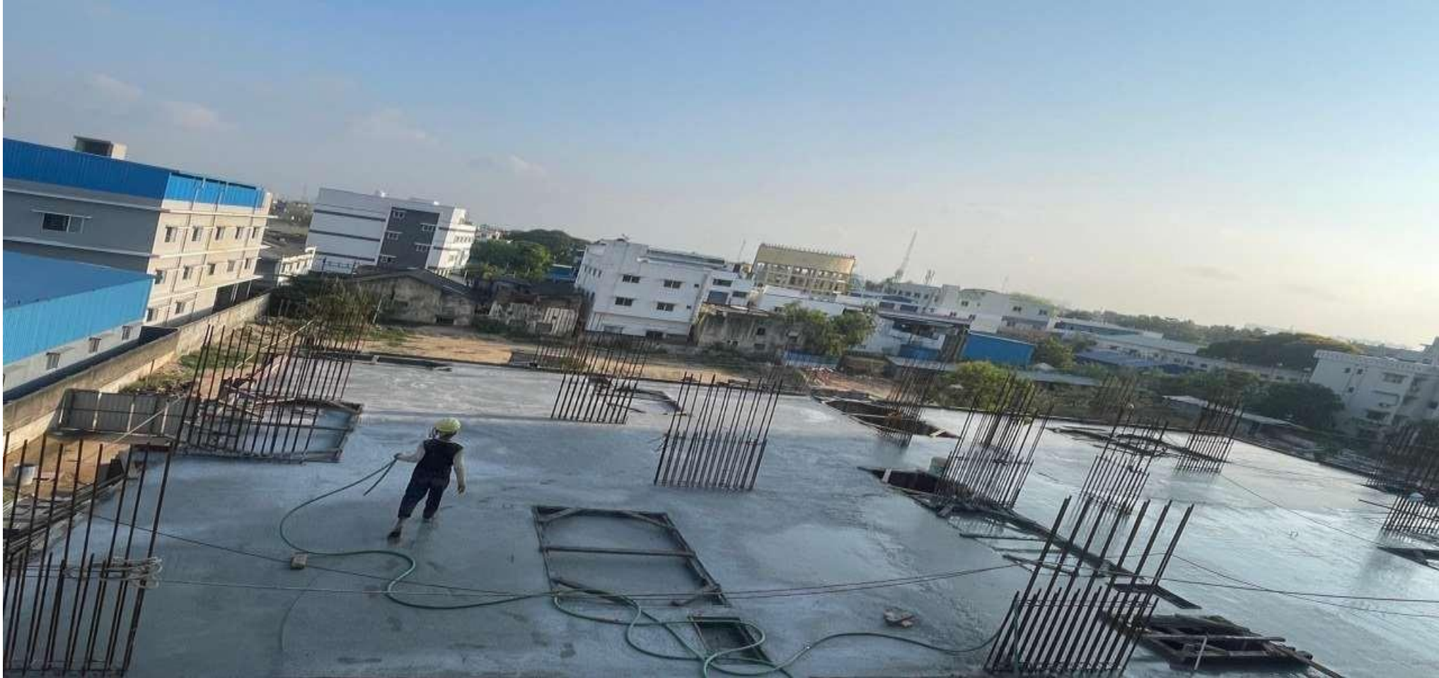
Pour 2 – 2 nd Floor roof slab concrete work completed.
