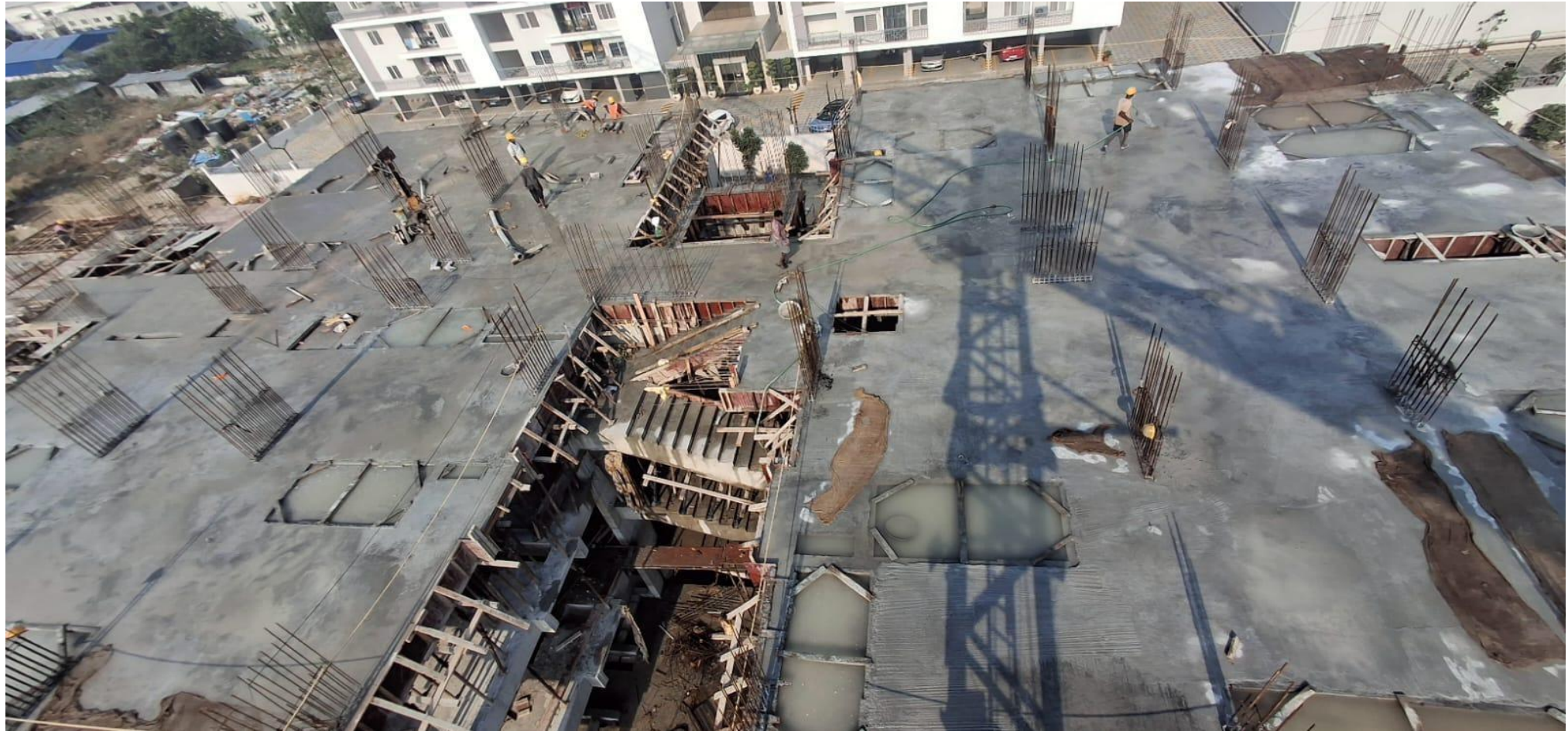
Pour 1 – 3 rd Floor roof slab concrete work completed.
