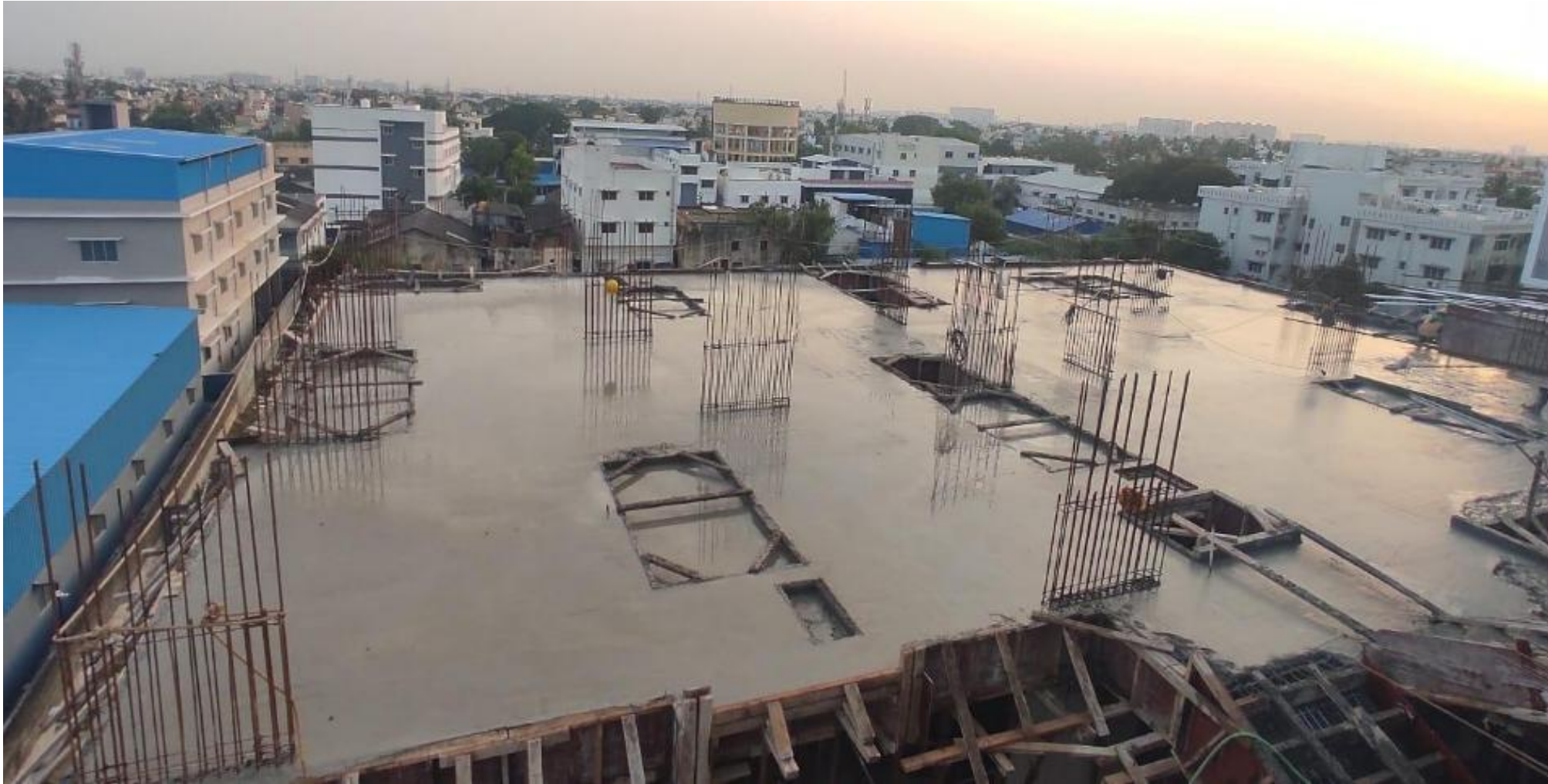
Pour 2 – 4 th floor roof slab concrete work completed.
