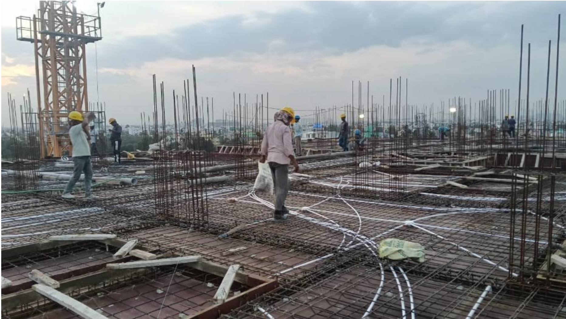
Pour 1 – 6 th Floor roof reinforcement work completed.
