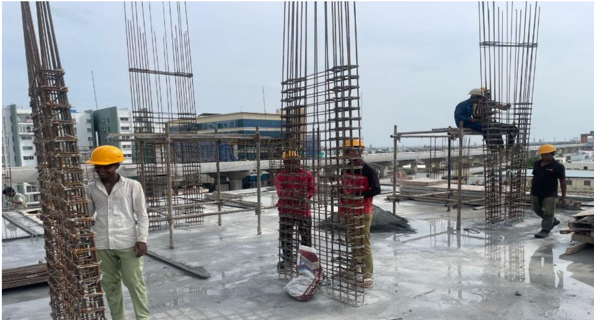
Pour 1 – 7 th Floor column reinforcement work in progress.
