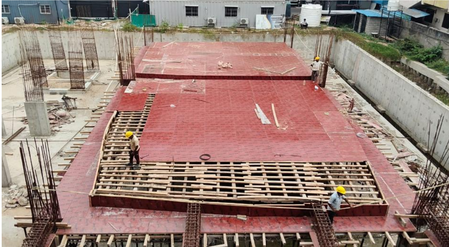
Tower 2 – Commercial basement roof shuttering work in progress.
