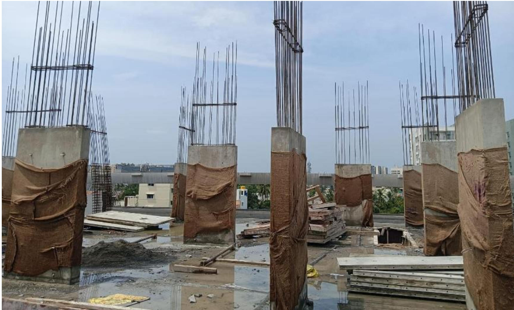
Pour 1 – 6 th floor column concrete work completed
