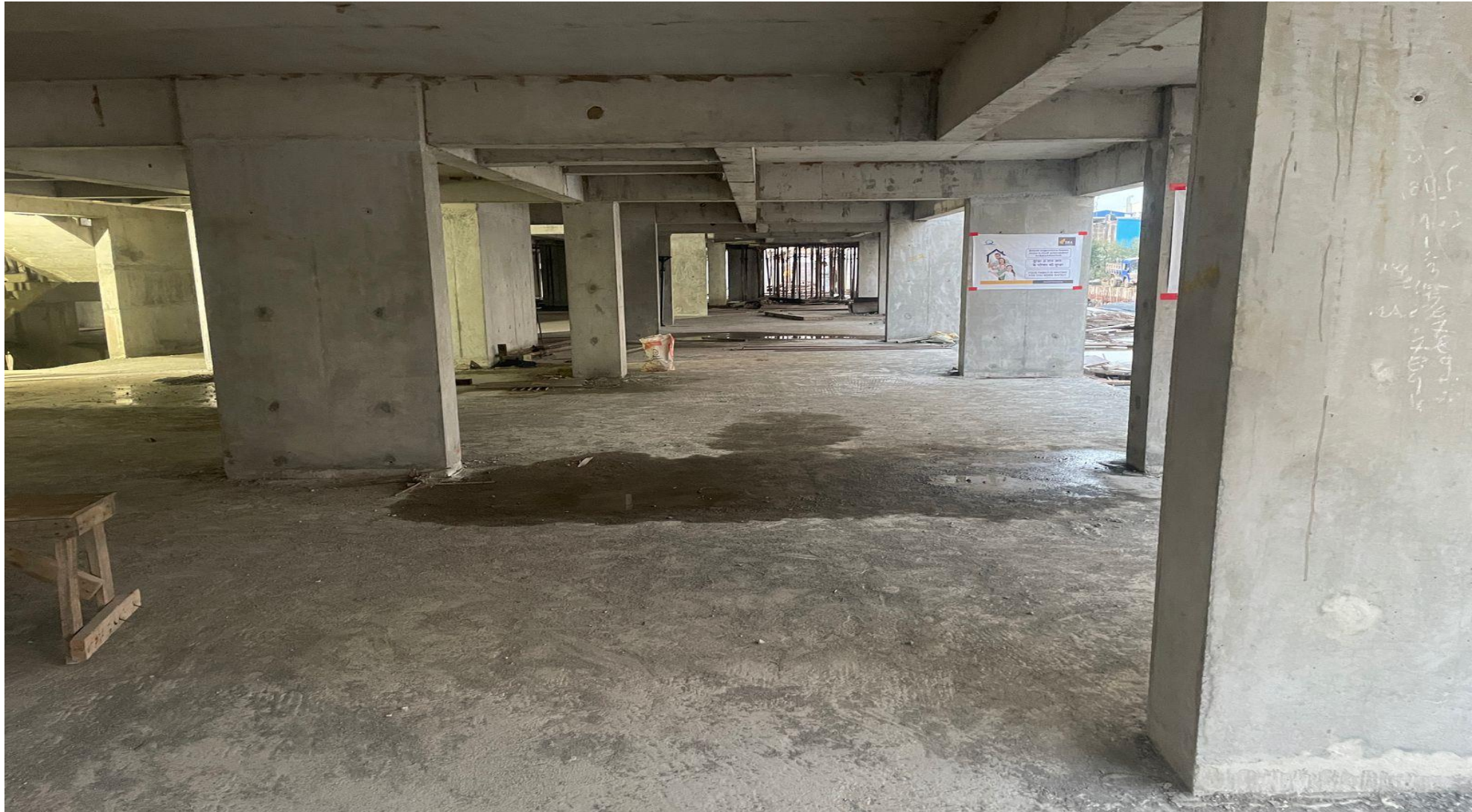
Pour-1 Stilt floor roof de-shuttering work completed .
