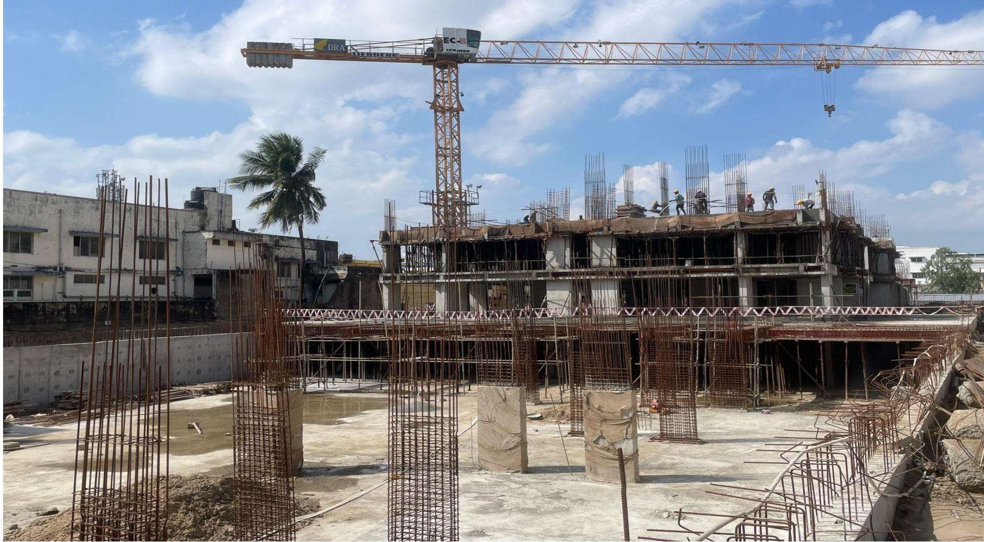
South east corner view.
