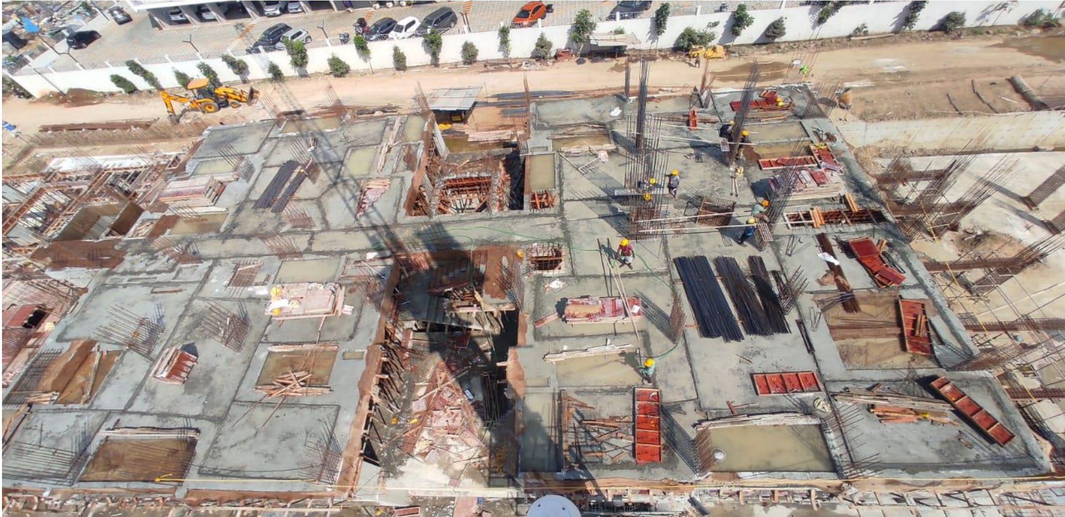
Pour-1 First floor roof slab concrete work completed.
