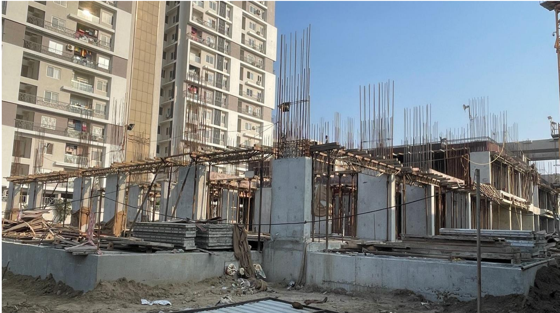
Northwest corner view.
