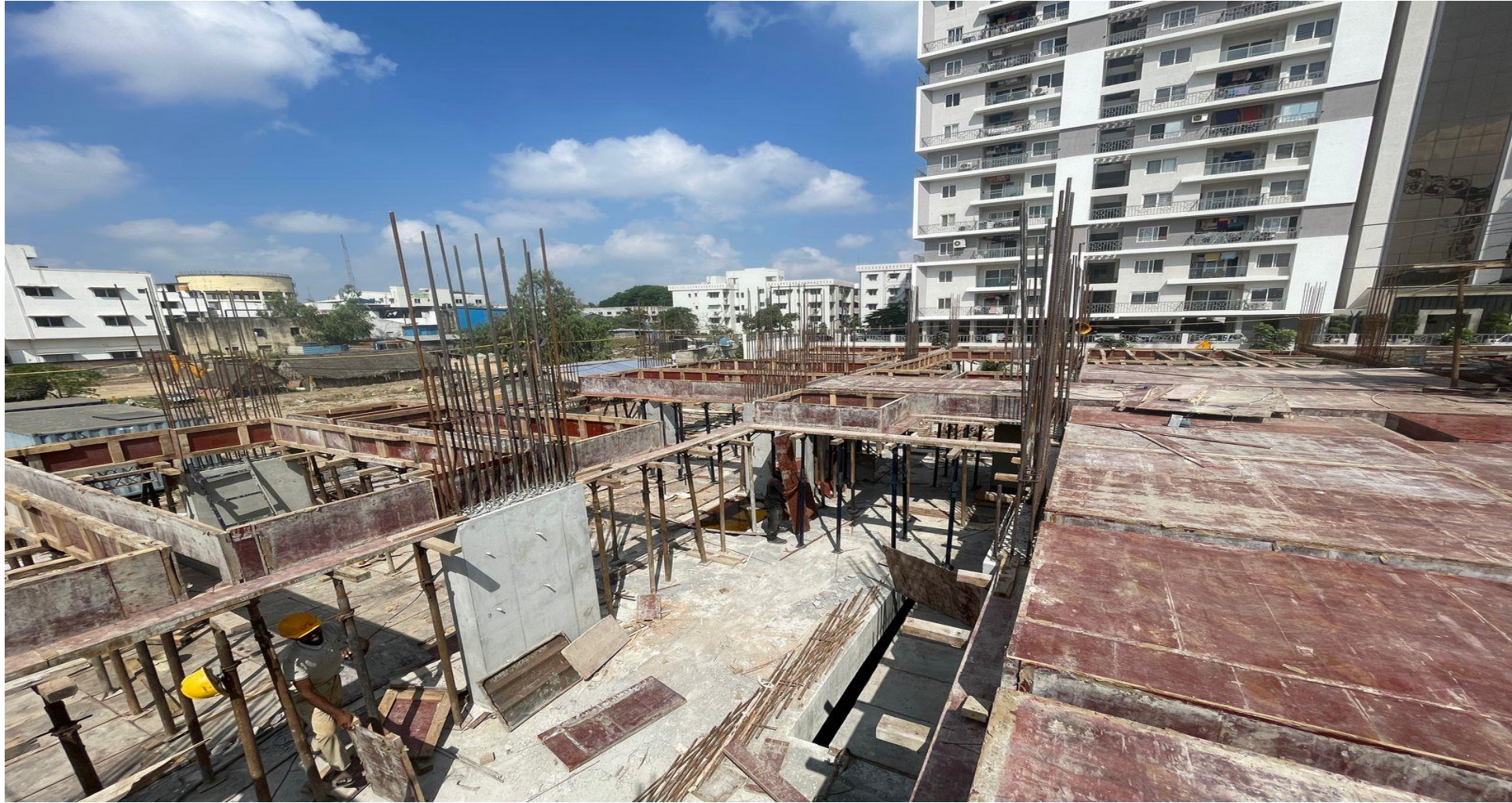
Pour-2 Stilt floor roof slab shuttering work in progress.
