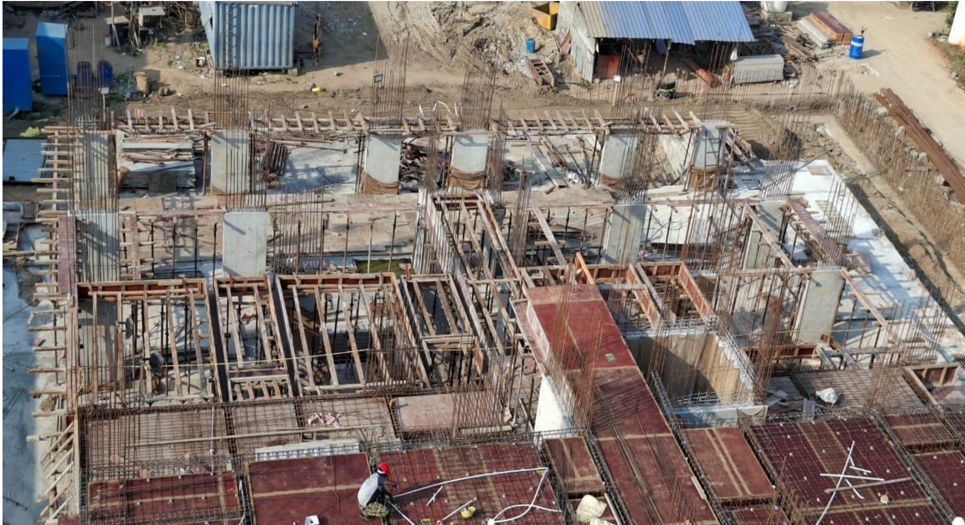
North Side View
