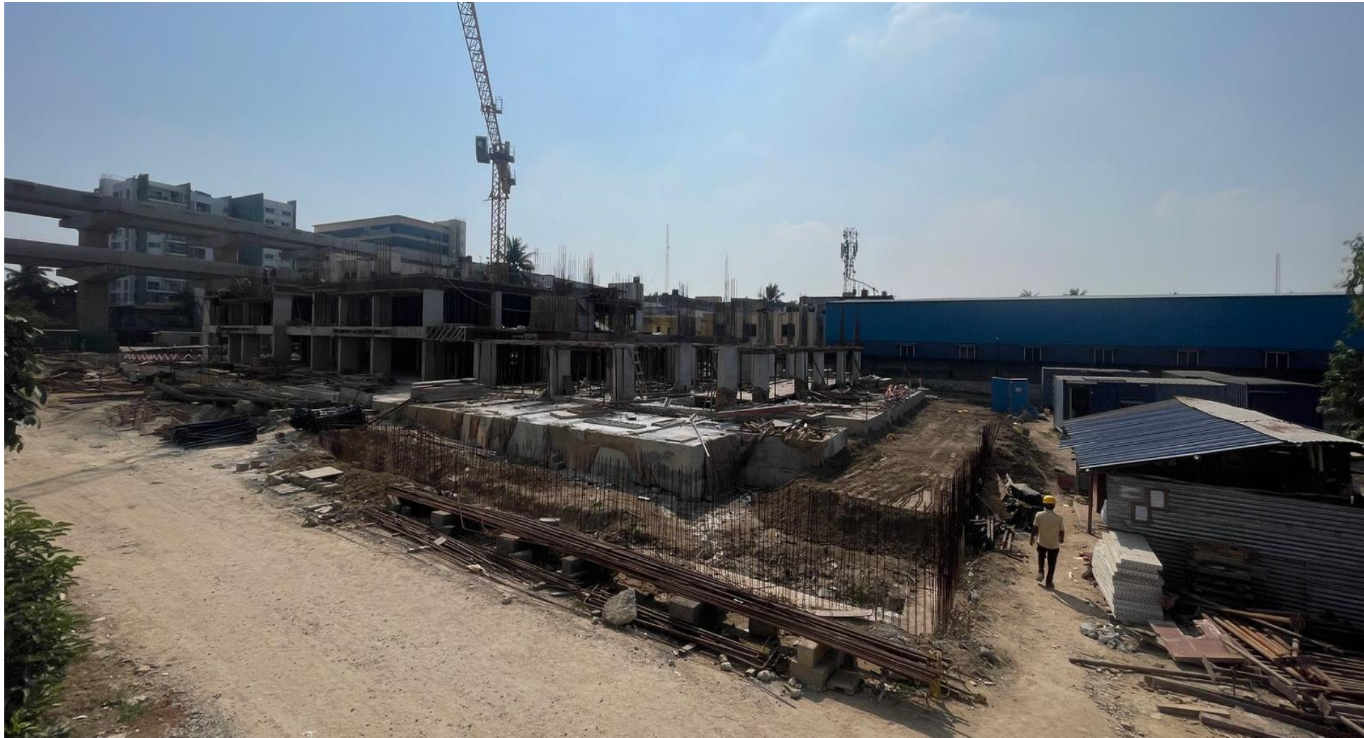
North east corner view.
