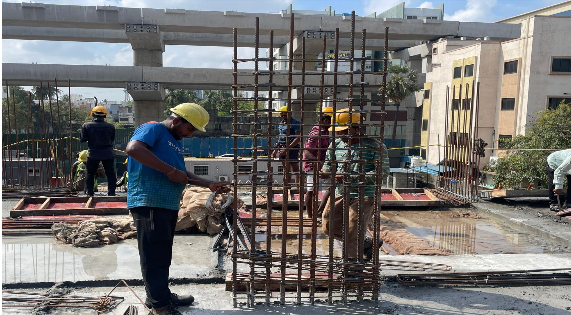
Pour-1 2 nd floor column reinforcement work in progress.
