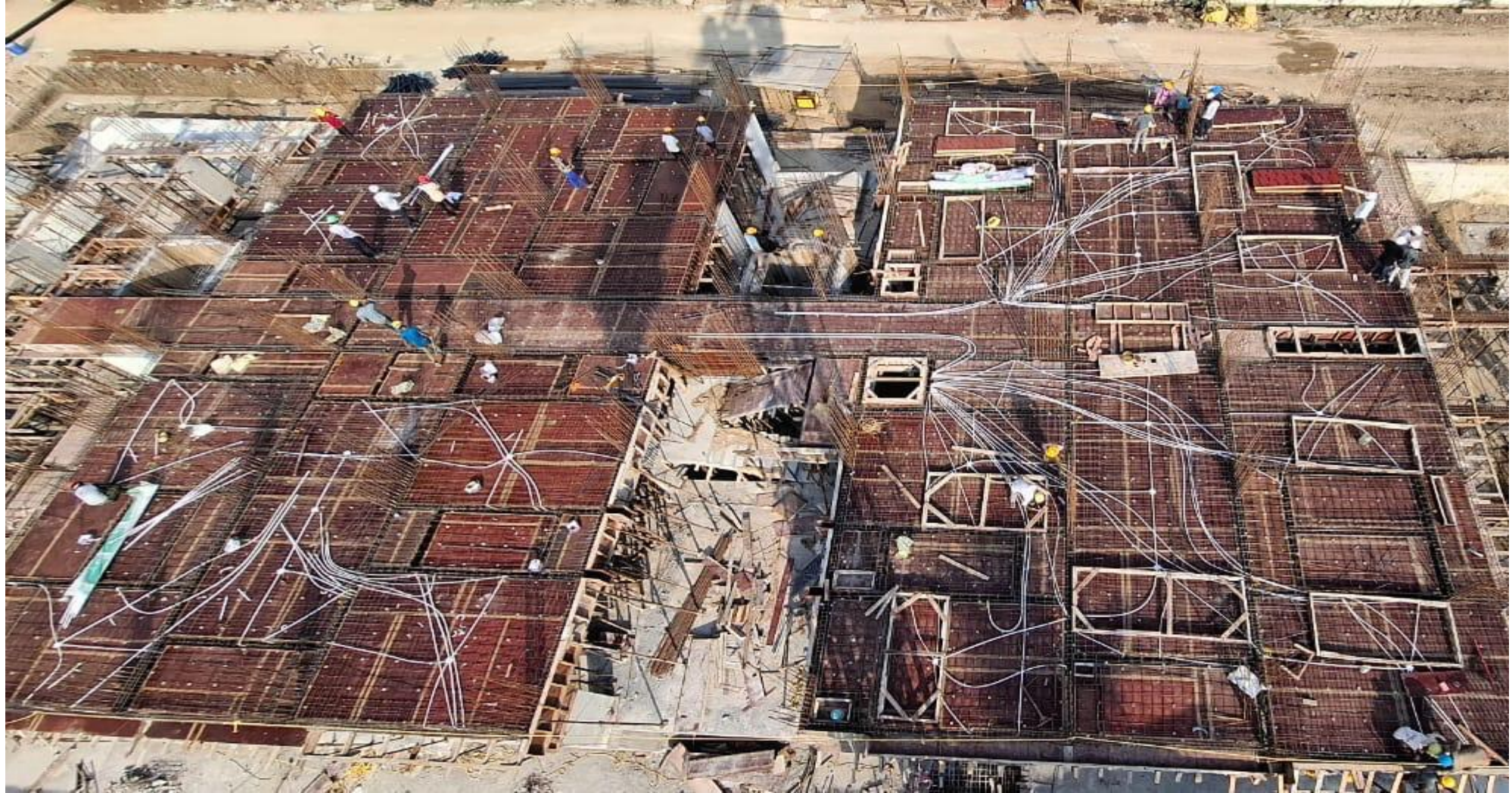
Pour-1 First floor electrical conduit pipe laying work completed.
