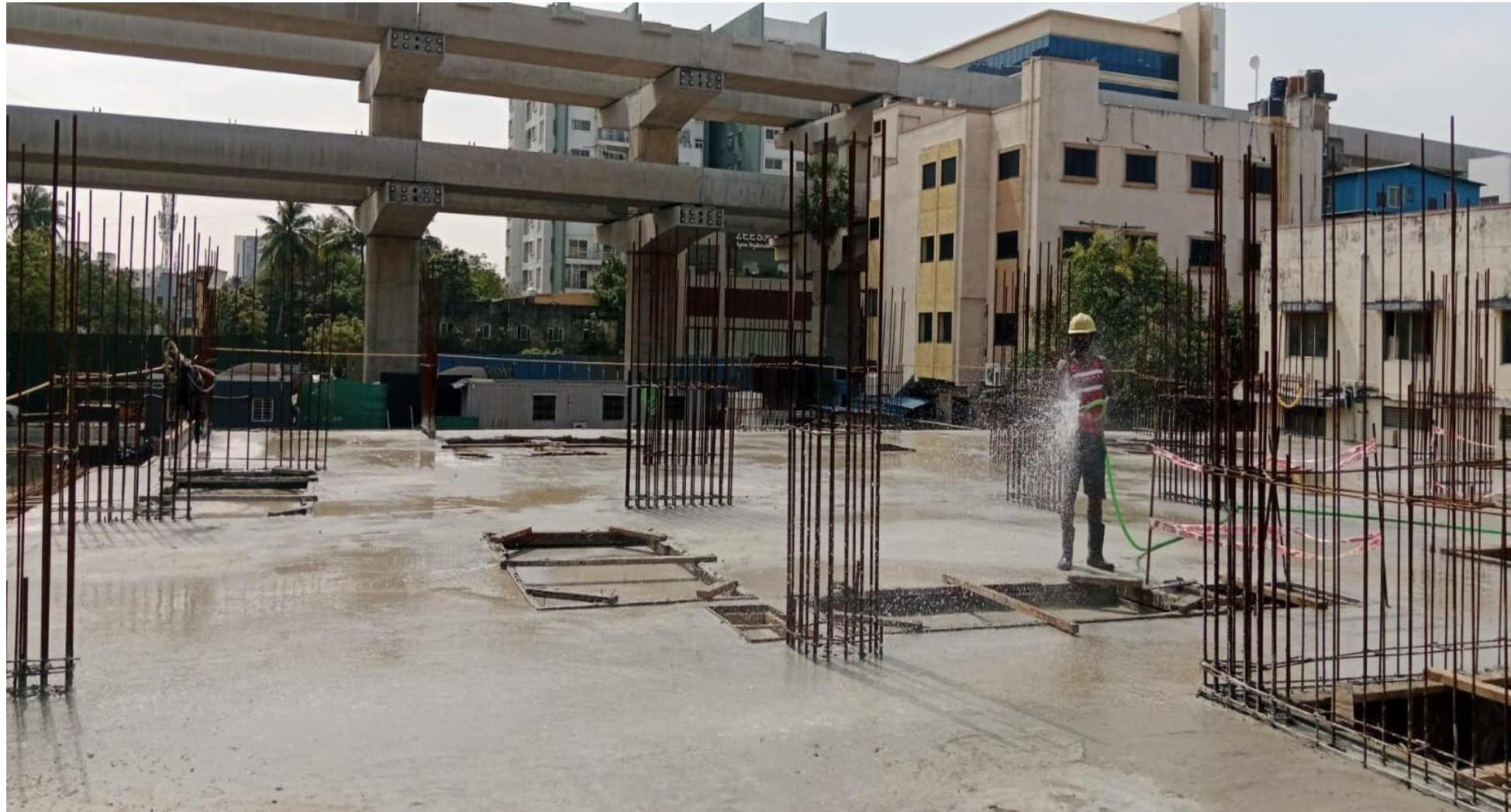
Stilt floor Pour-01 roof slab initial curing work completed.
