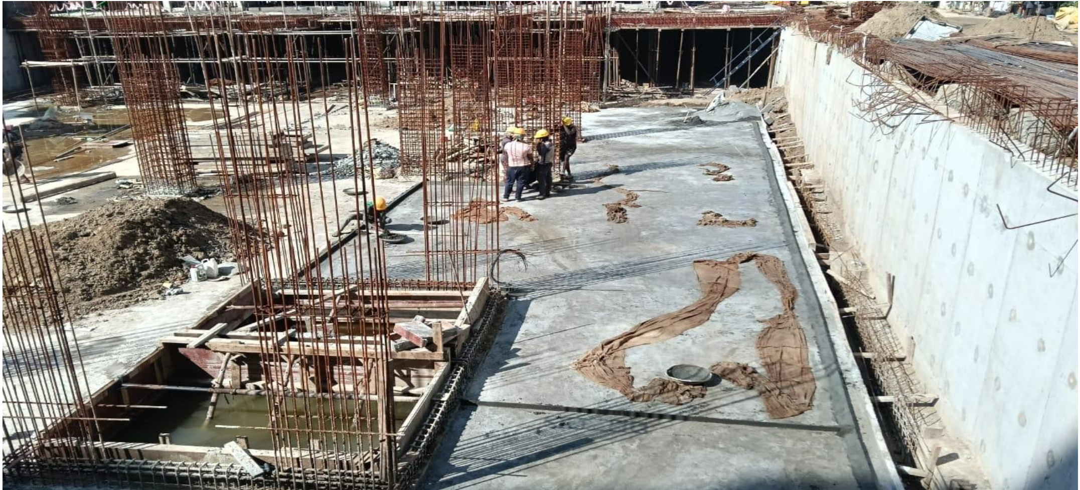
T-2 Pour-03 commercial area grade concrete work completed.
