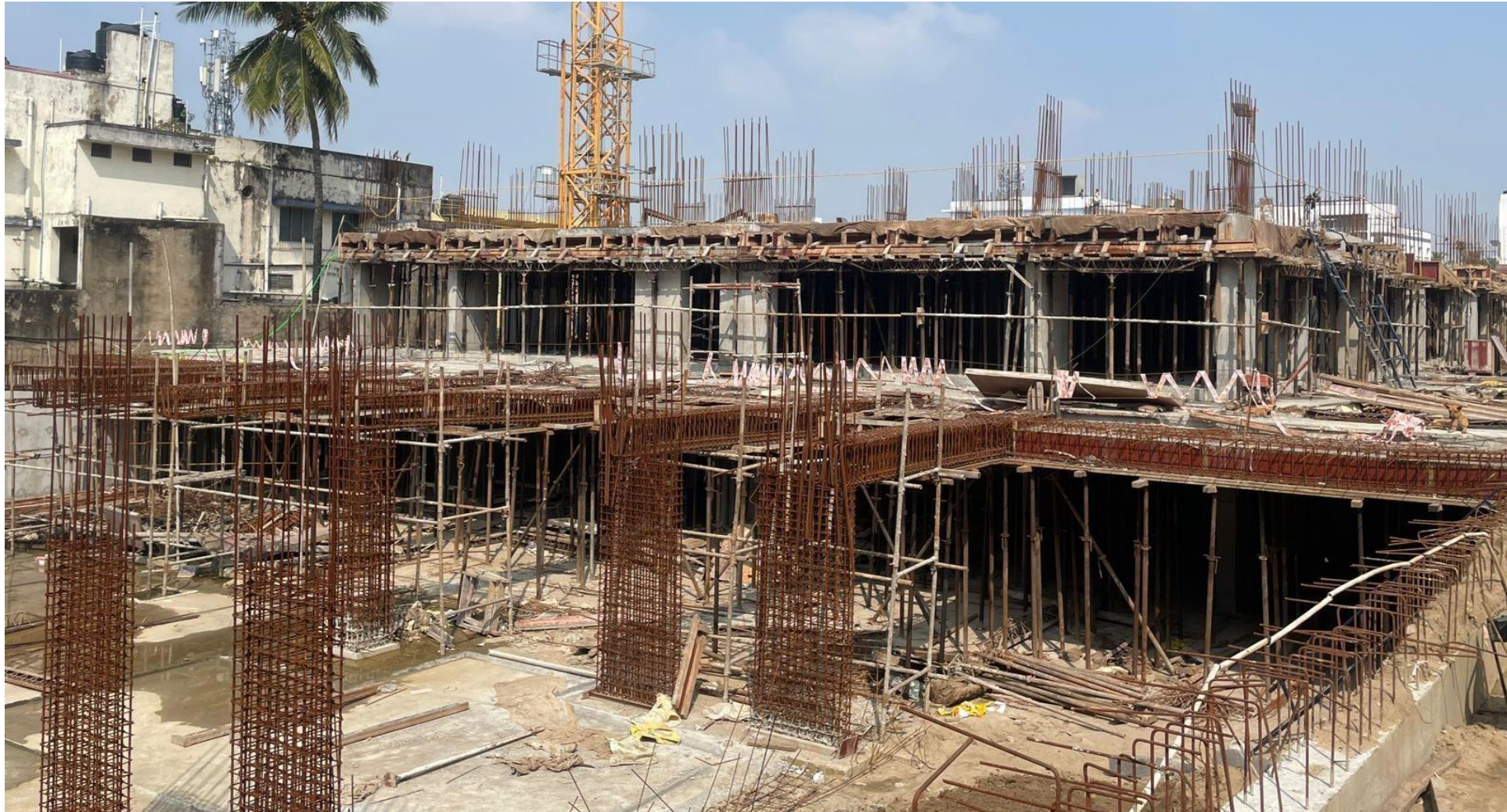
North east corner view.
