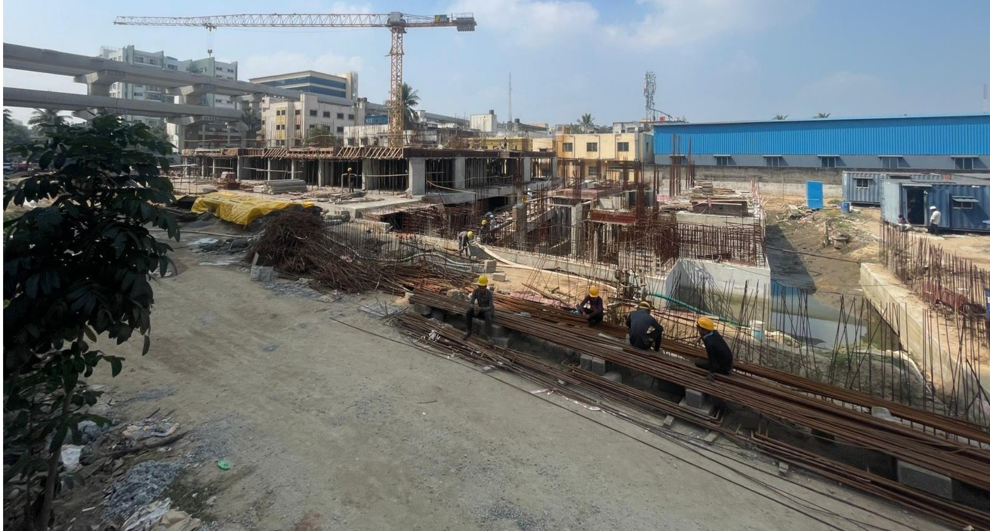
South east corner view.
