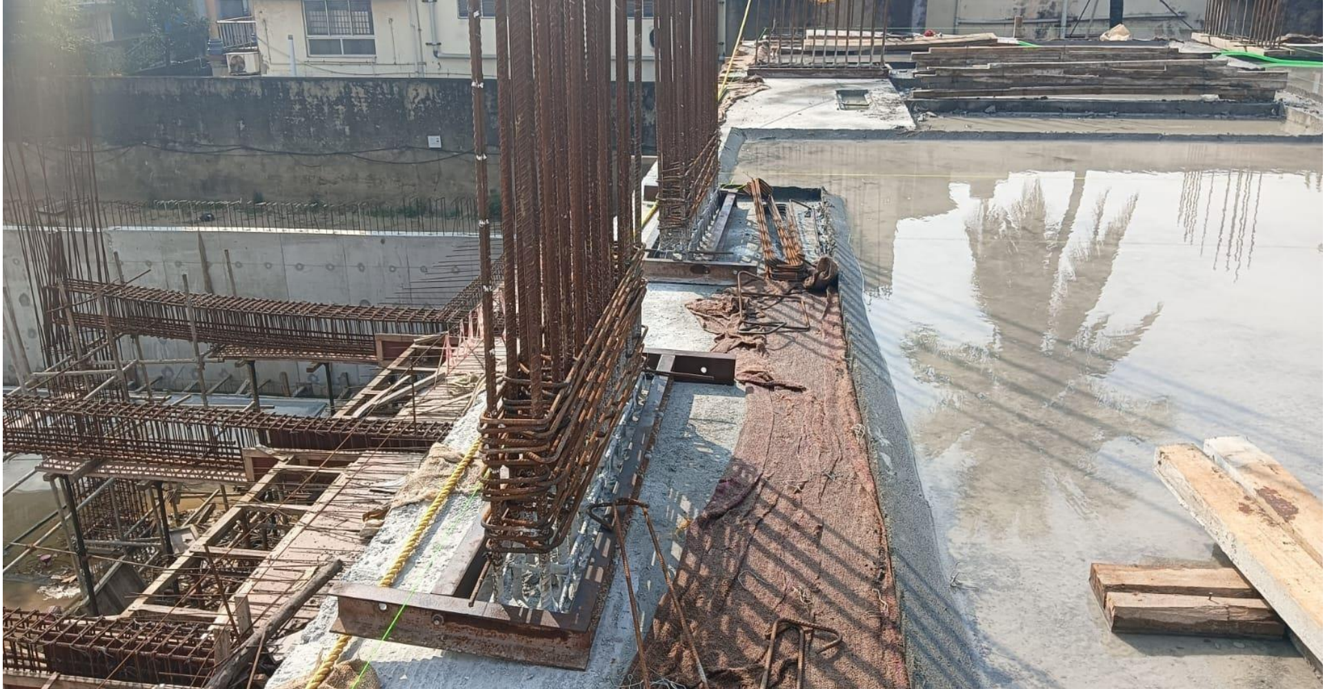
Pour-3 first floor column starter fixing work in progress.
