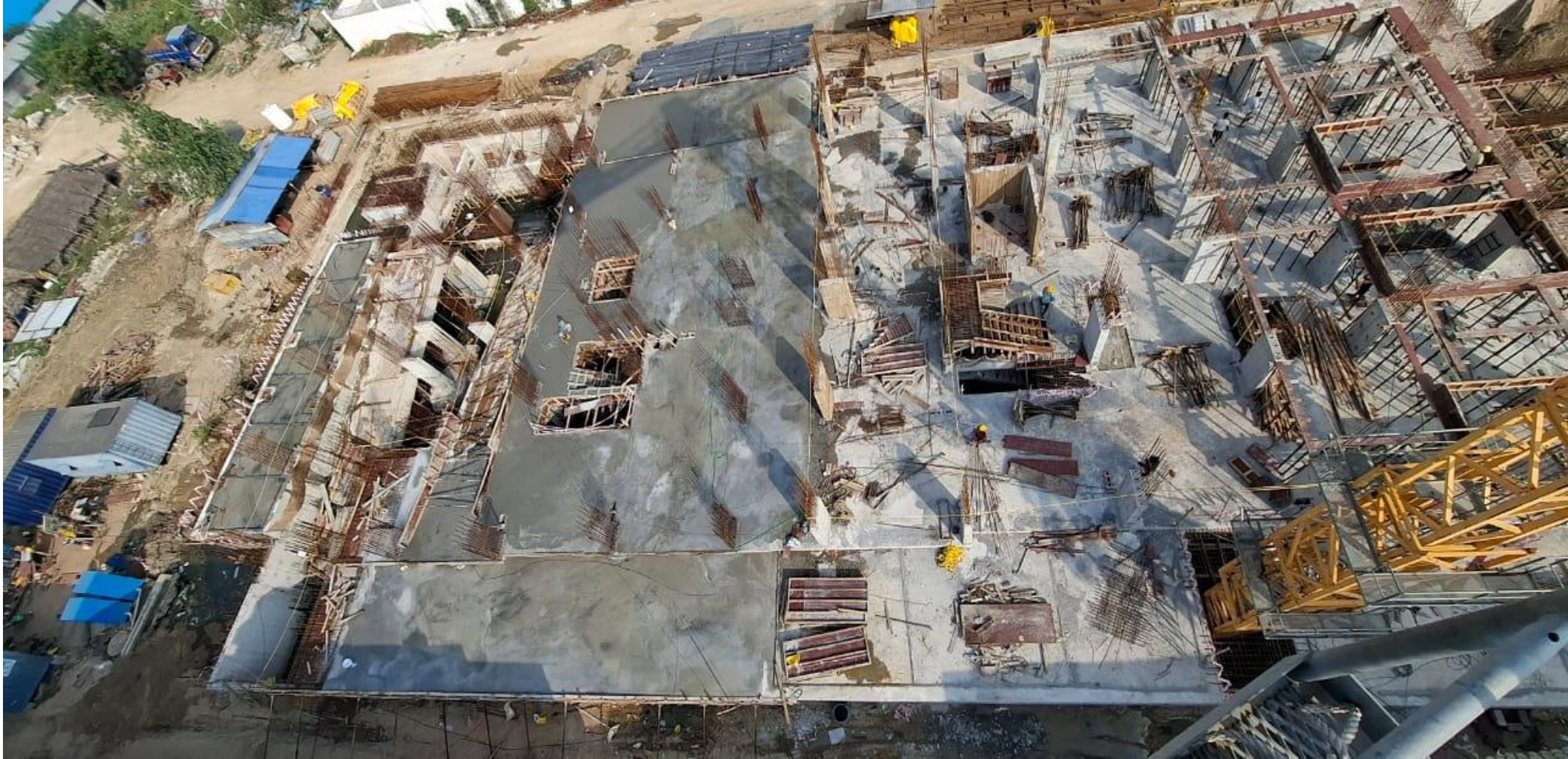
Pour-2 basement roof slab concrete work completed.
