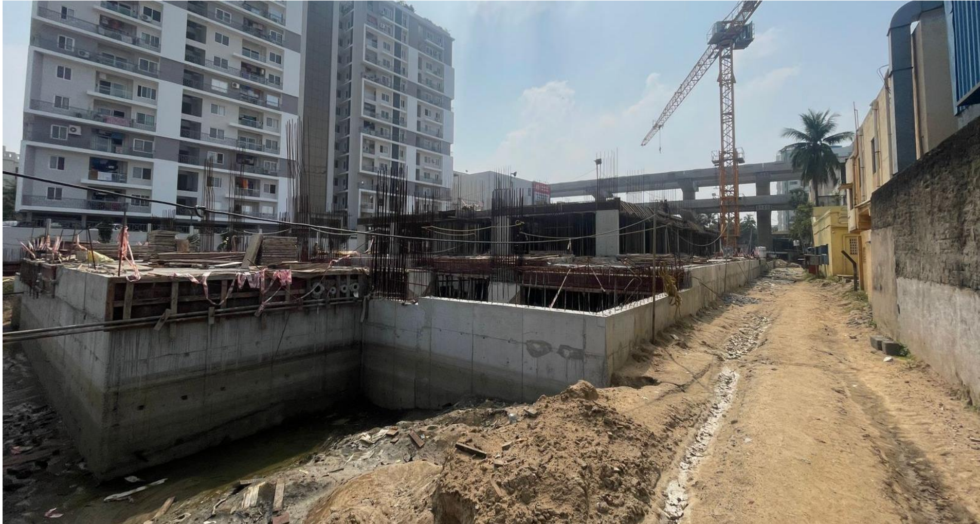
Northwest corner view.
