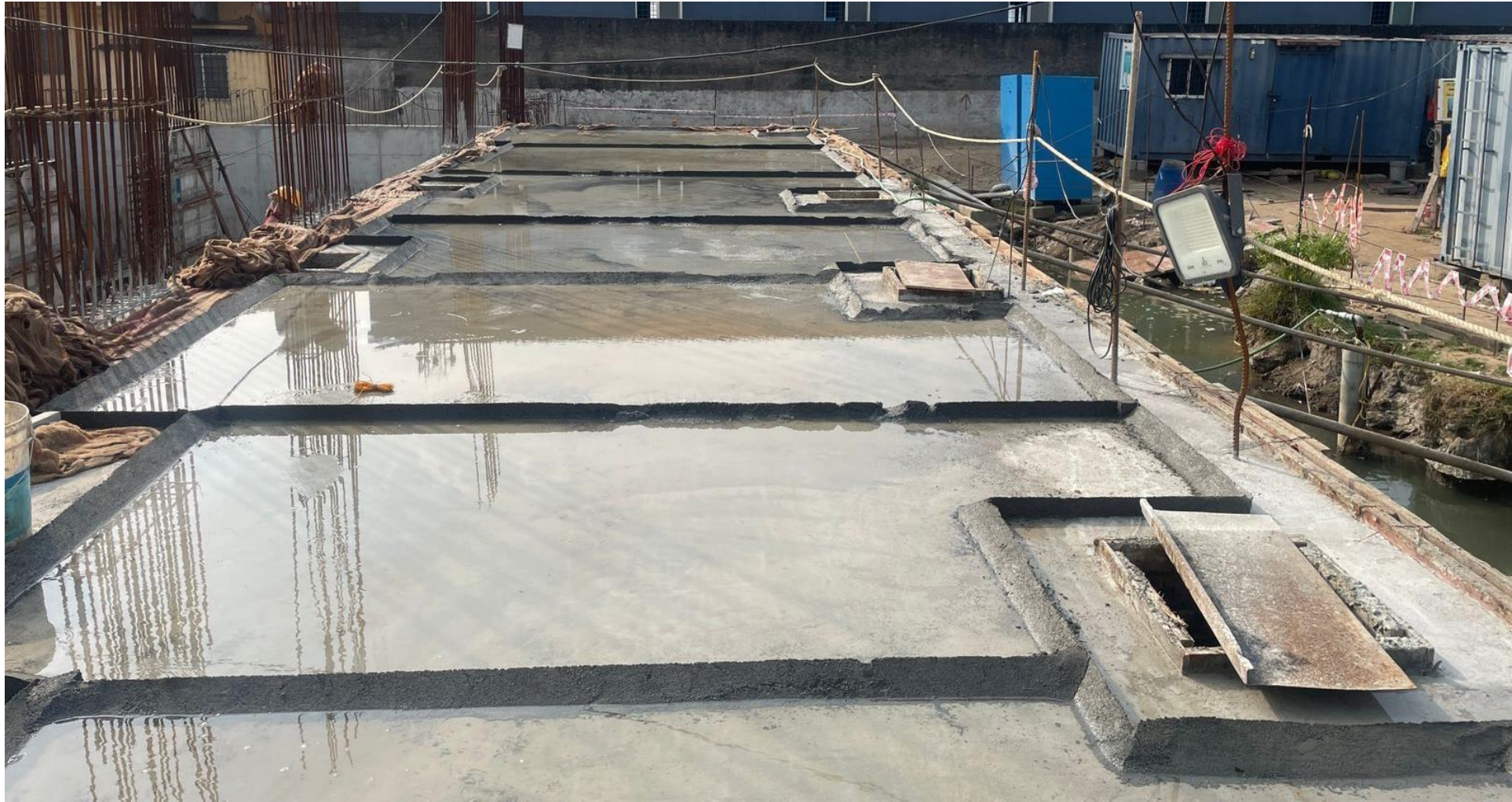
UG sump cover slab curing work in progress.
