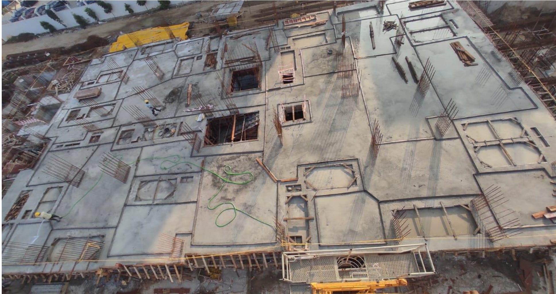
Pour-1 stilt floor roof slab curing work in progress.
