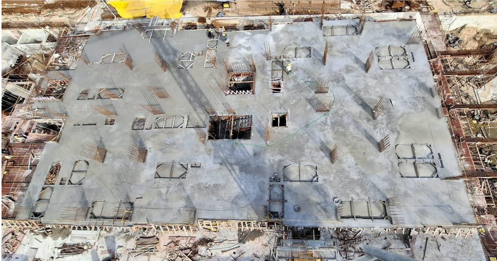
Pour-2 stilt floor roof slab concrete work completed.
