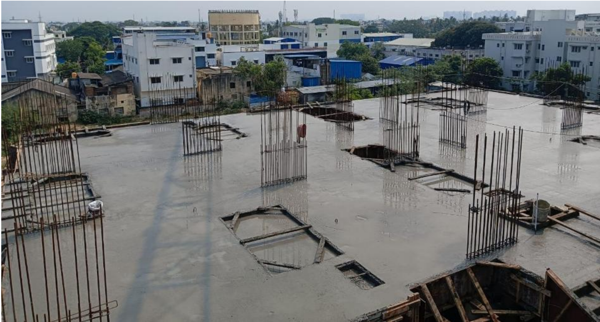
Pour 2 – 3 rd floor roof slab concrete work completed.
