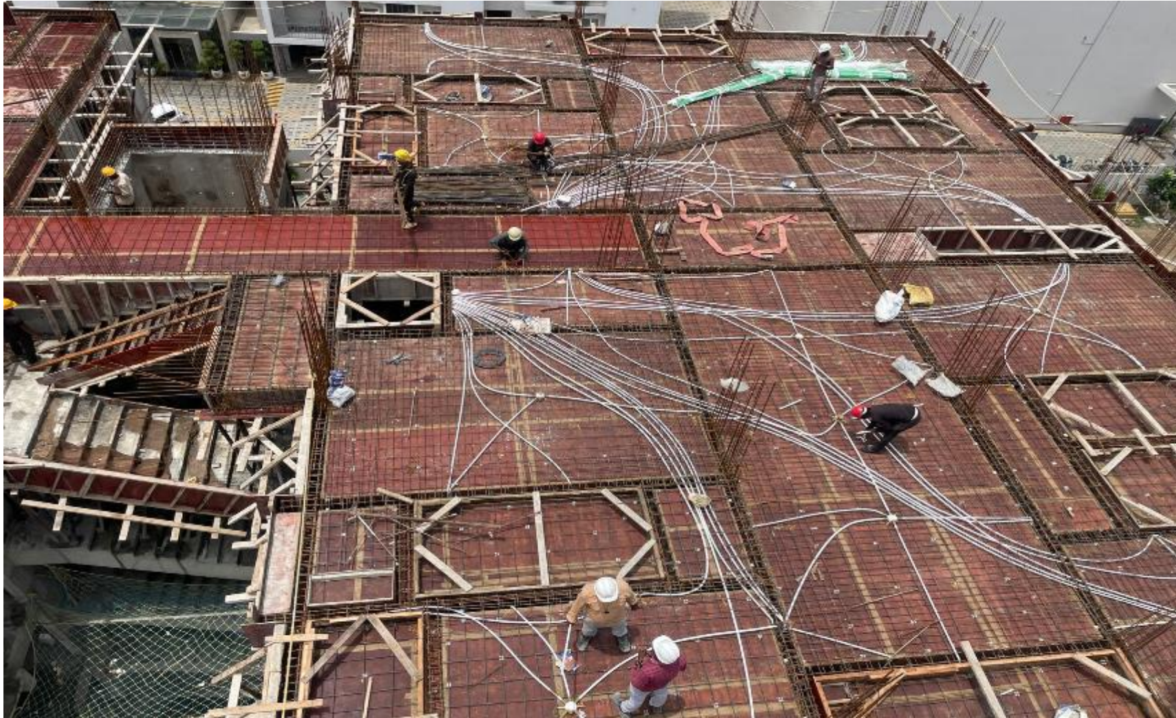
Pour 1 – 5 th floor roof slab electrical conduit laying work completed.
