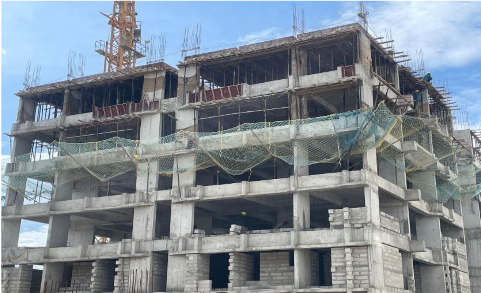
Safety catch net installation work.
