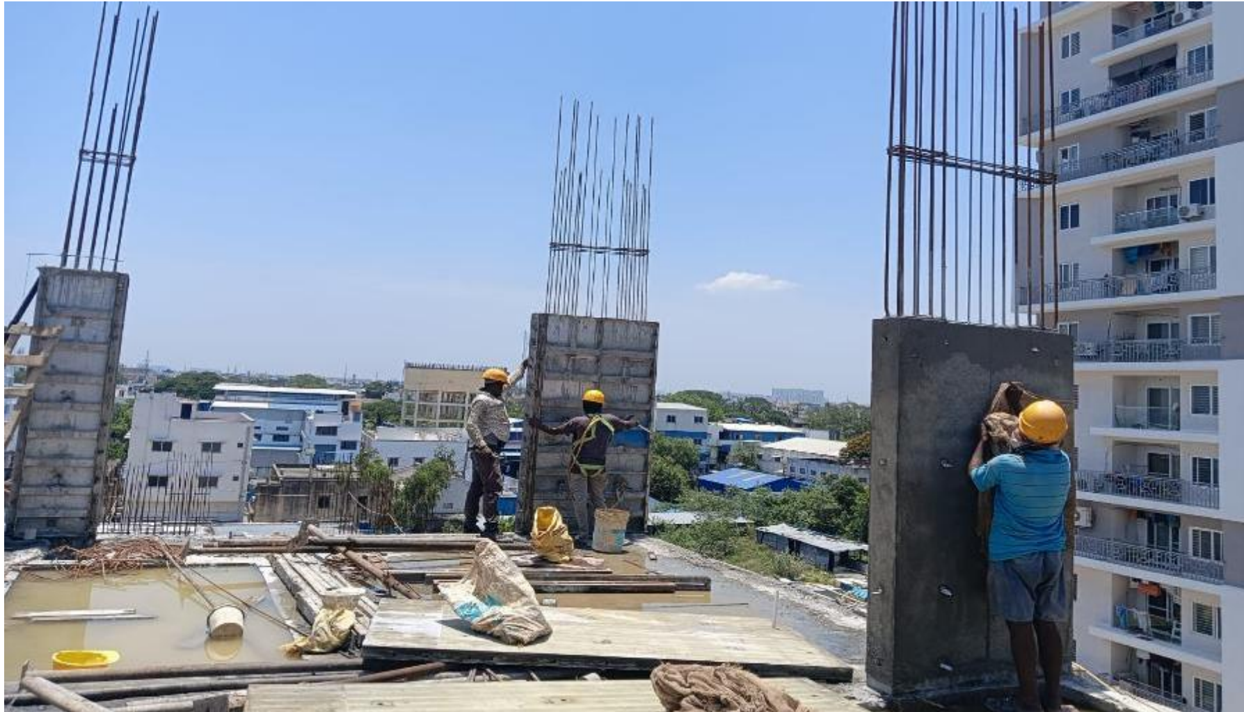
Pour 1 – 5 th floor column concrete work completed.
