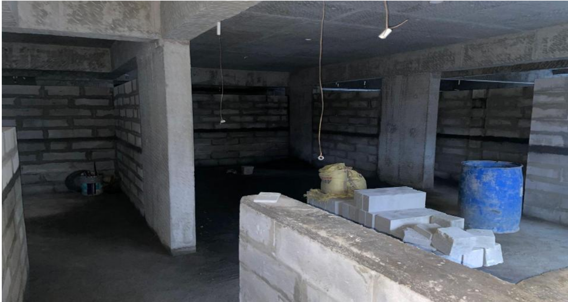
1 st Floor block work in progress
