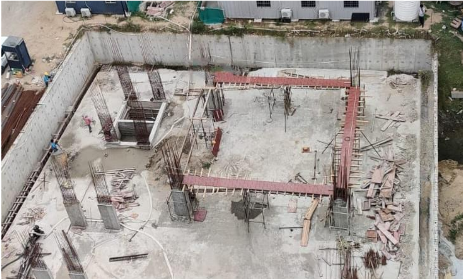
T2 pour-1 basement roof PT beam shuttering work commenced.
