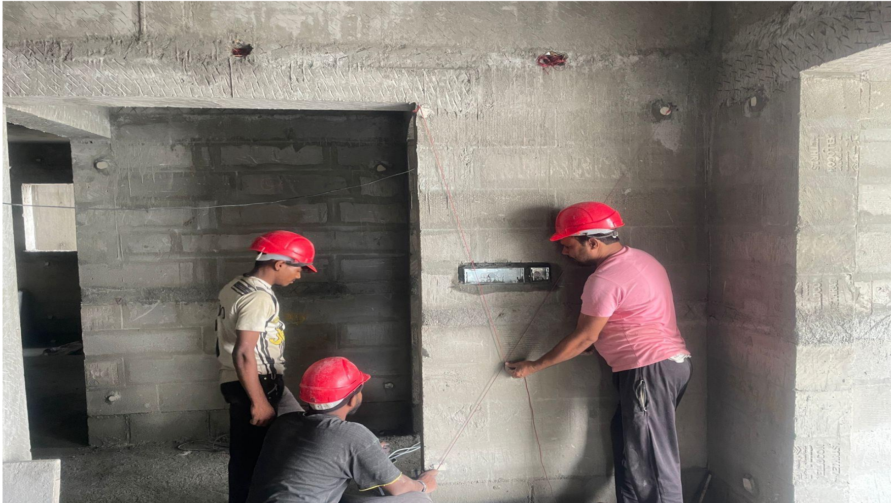
First floor electrical metal box fixing work in progress.
