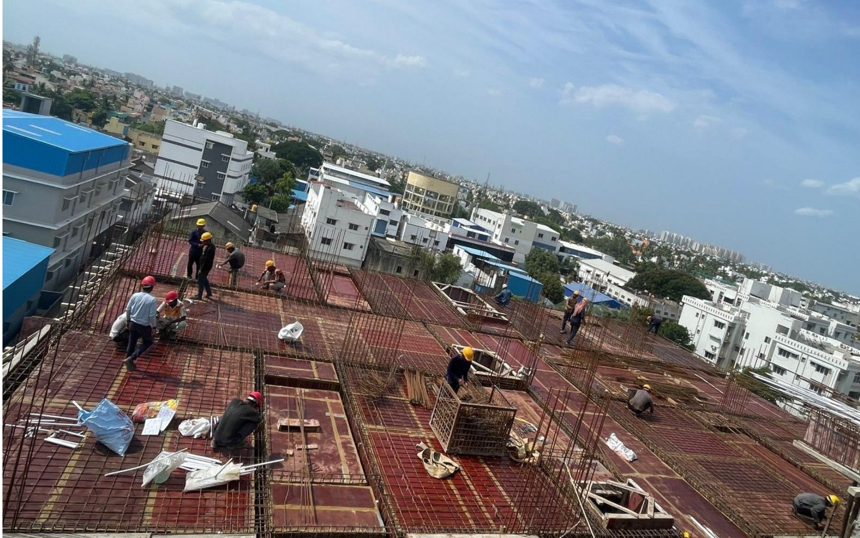
Pour 2 – 5 th Floor roof shuttering work completed.
