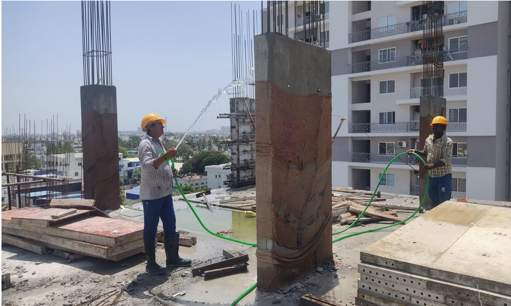
Pour 1 – 7 th floor column curing work in progress.
