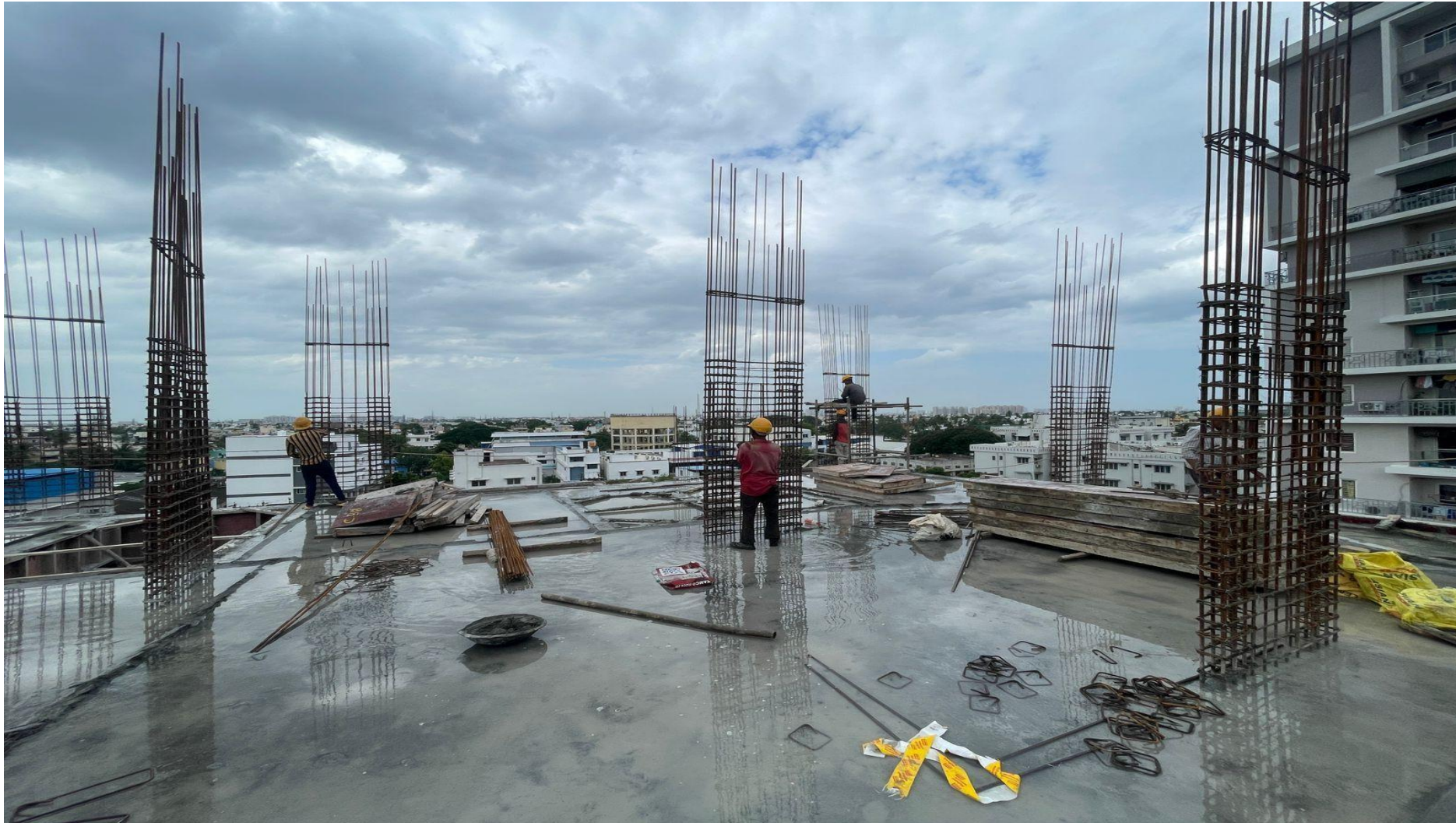
Pour 2 – 6 th Floor column reinforcement work completed (22/22) .
