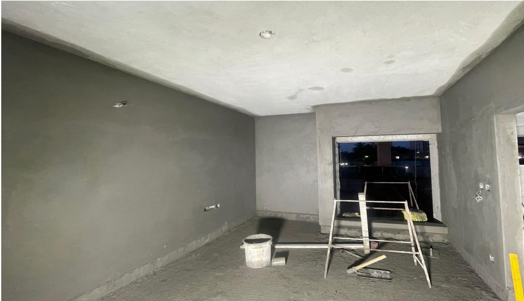
First floor wall plastering work in progress.
