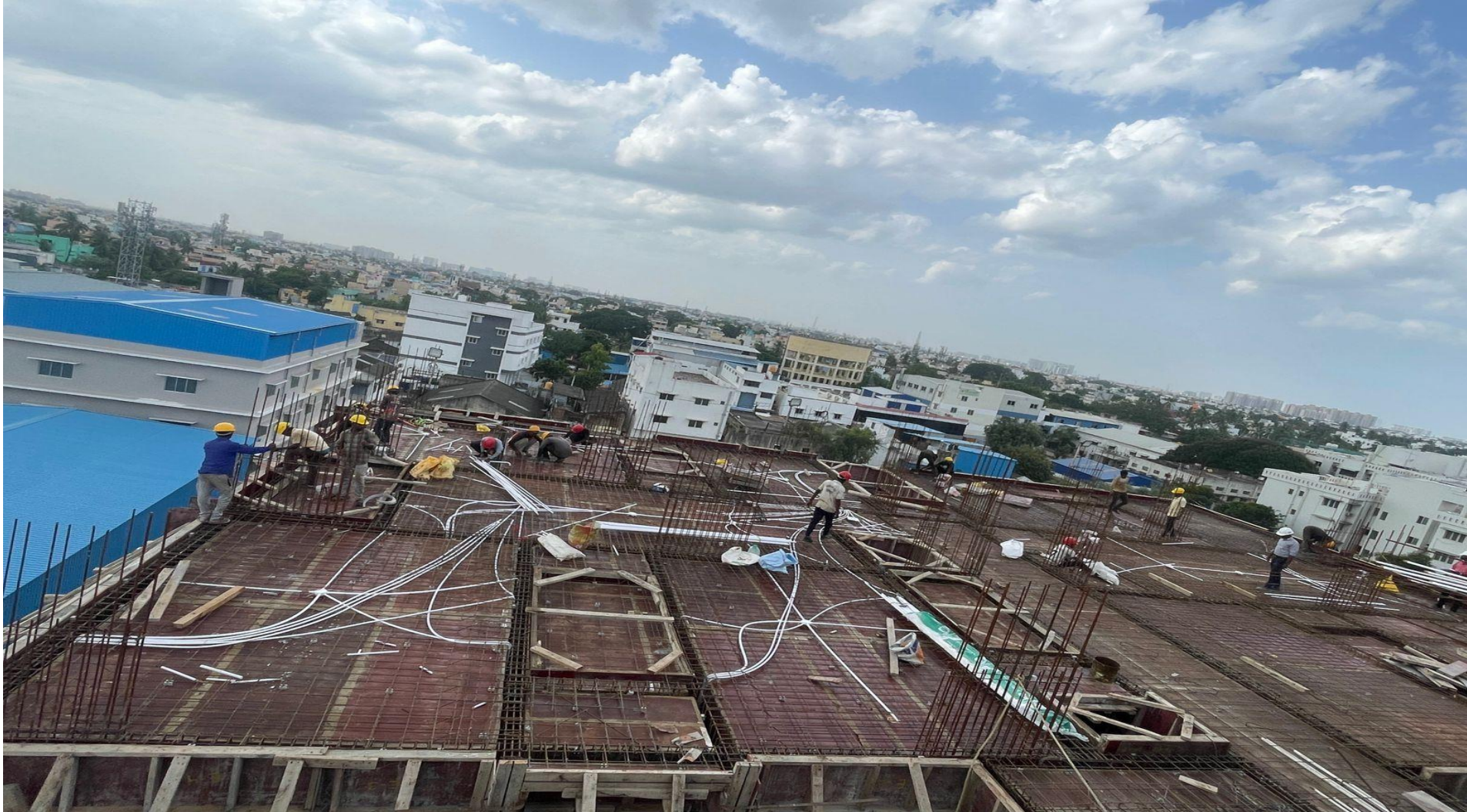
Pour 2 – 5 th Floor roof reinforcement work completed.
