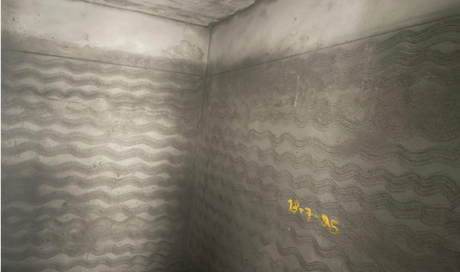
First floor toilet wall plastering work in progress.
