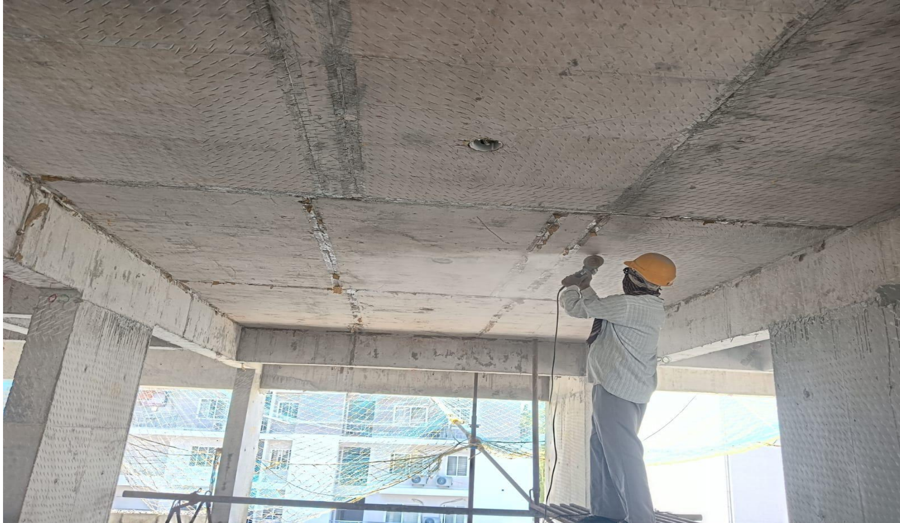
Fifth floor hacking work in progress.
