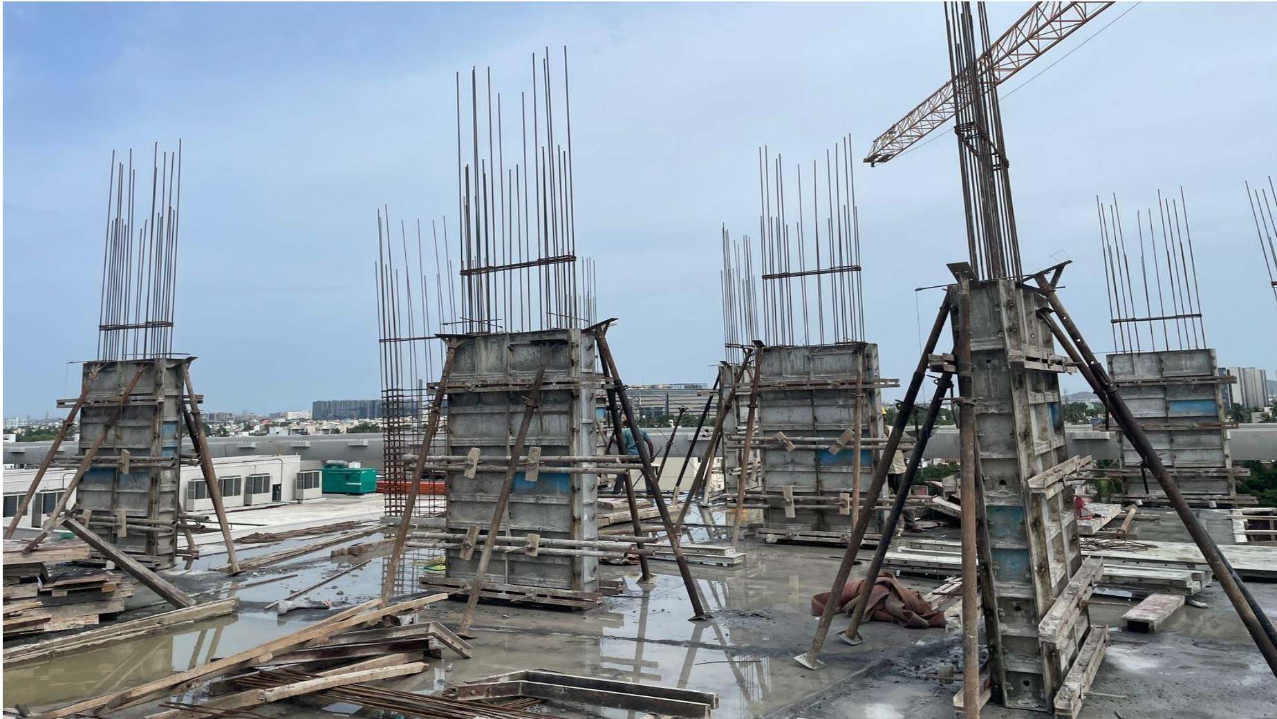
Pour 1 – 7 th floor column fixing work completed (45/45).
