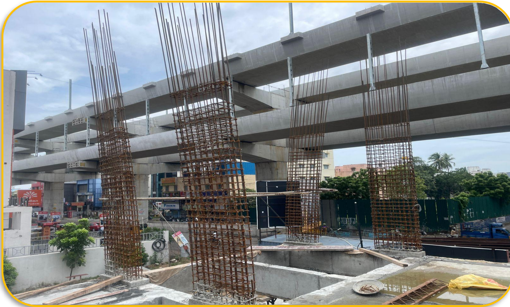
Tower -2 first floor column reinforcement work completed .
