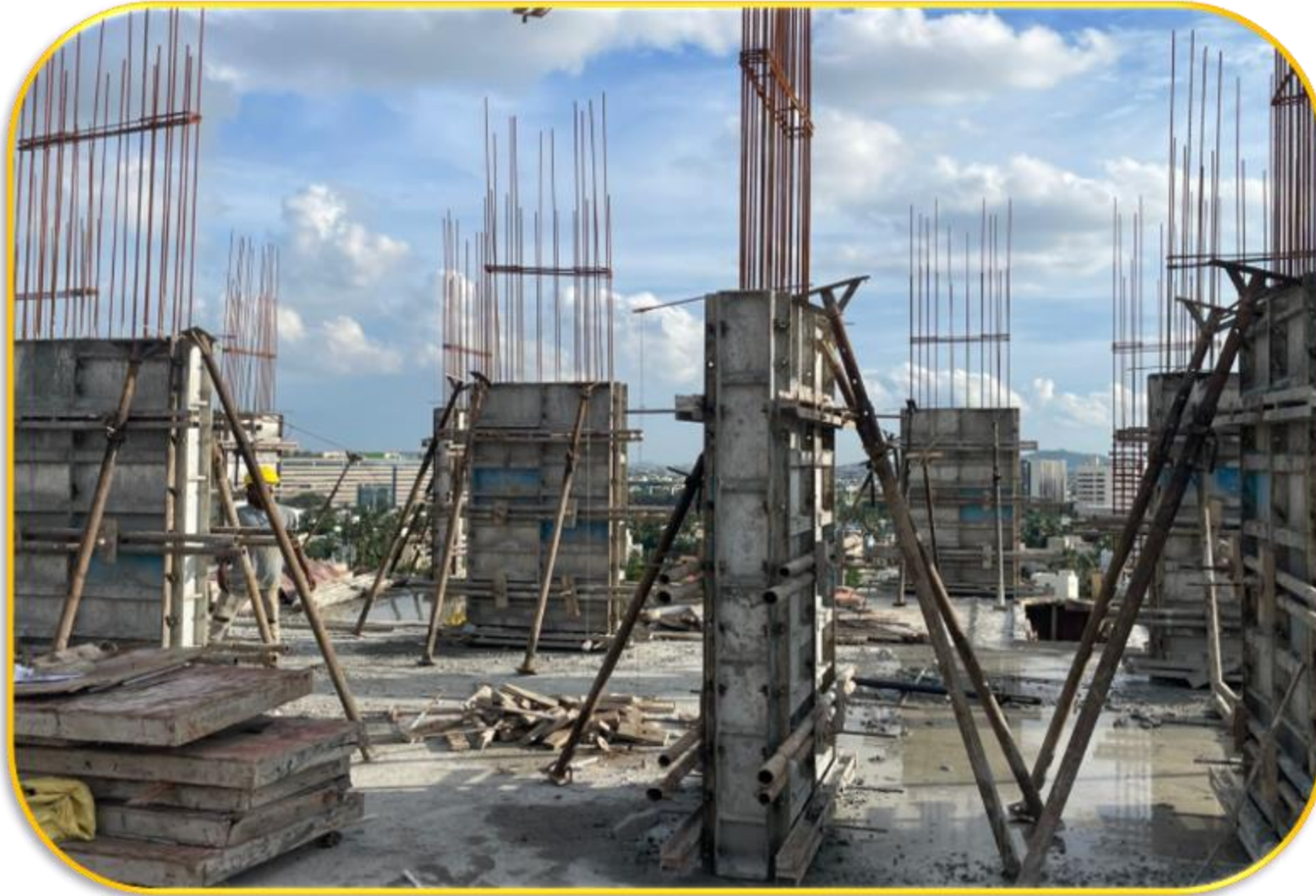
Pour 1 – 12 th floor column shuttering work in progress.
