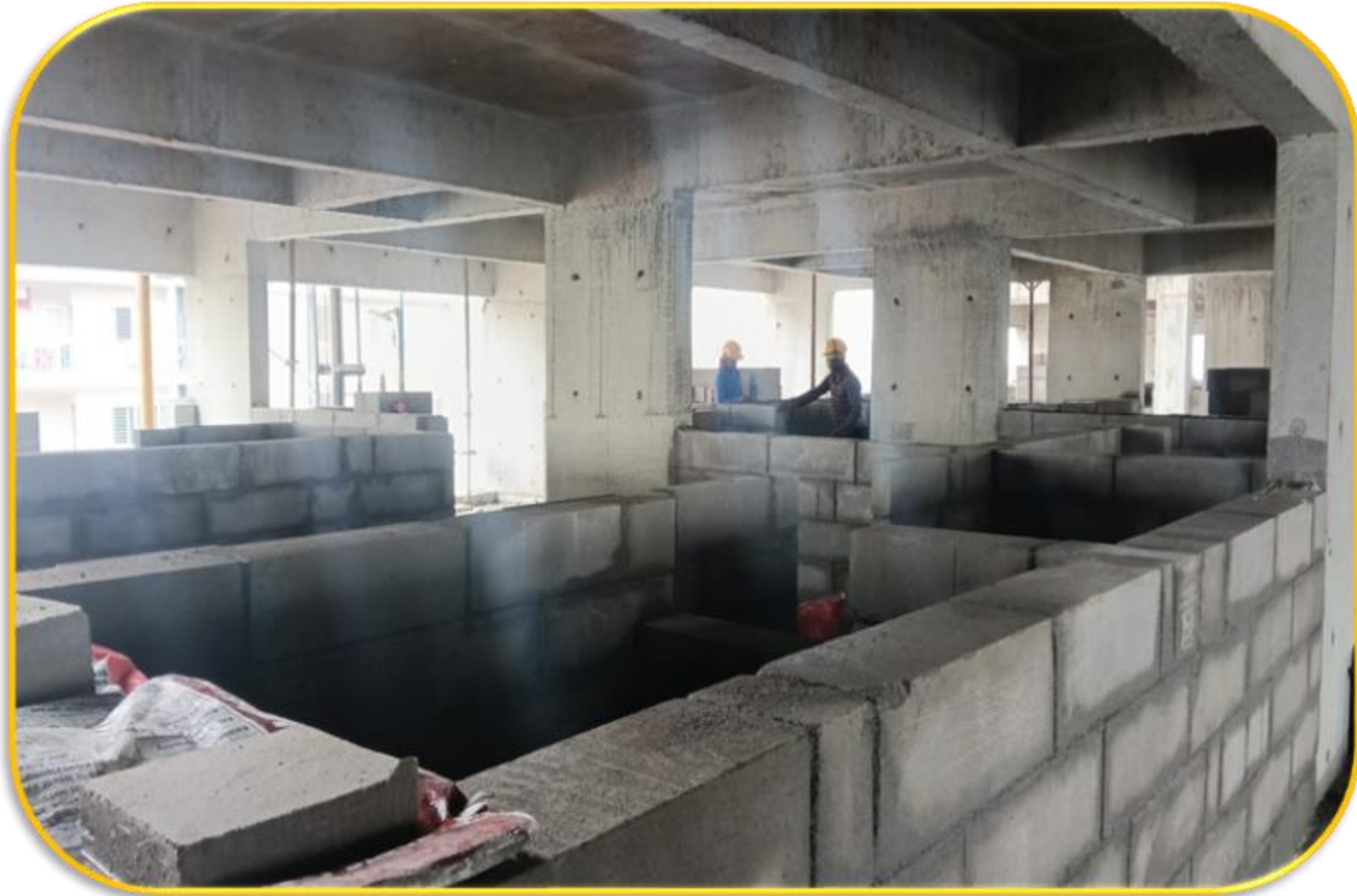
9 th Floor block work in progress.
