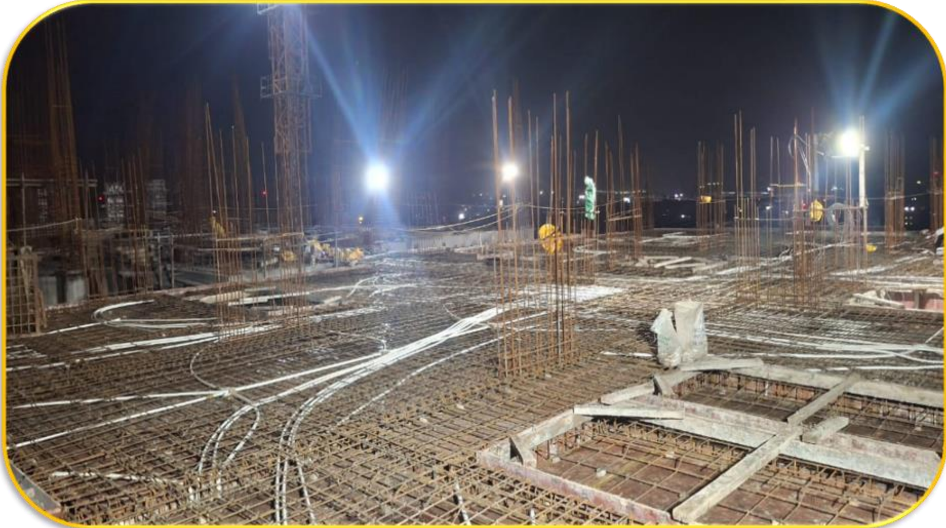
Pour 2 – 11 th Floor roof reinforcement work completed.
