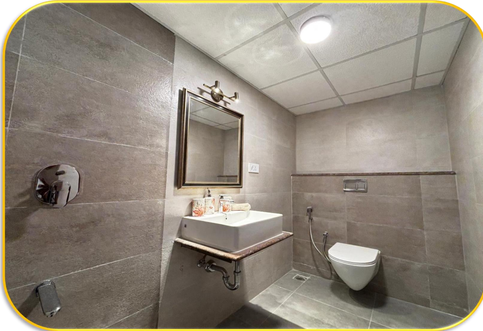
BED ROOM 2 TOILET
