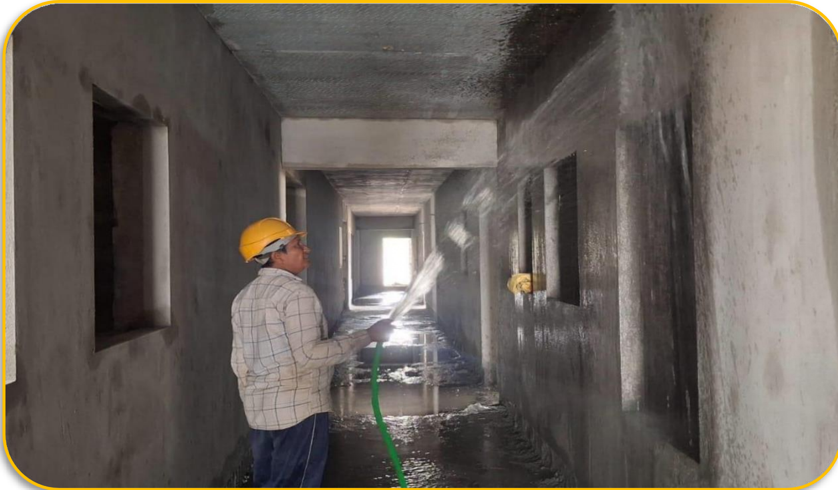
1 st floor corridor plastering work completed.
