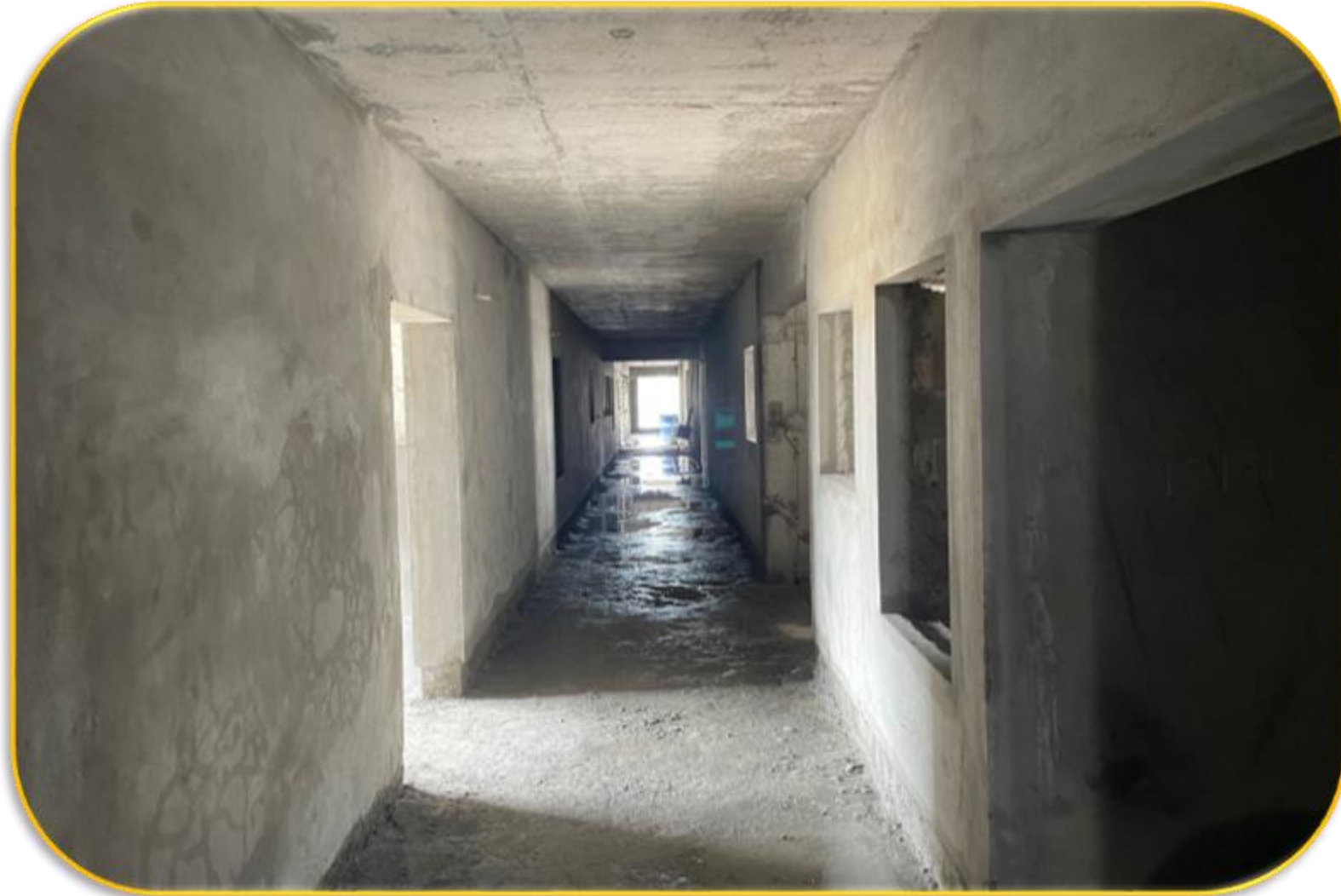
2 nd Floor corridor inner plastering work completed.
