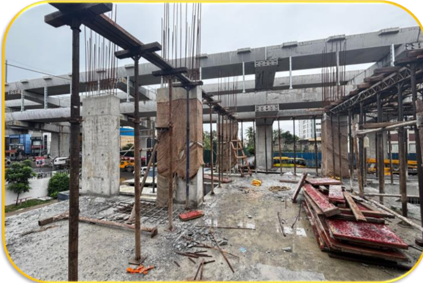
Tower 2 1 st floor column concrete work completed
