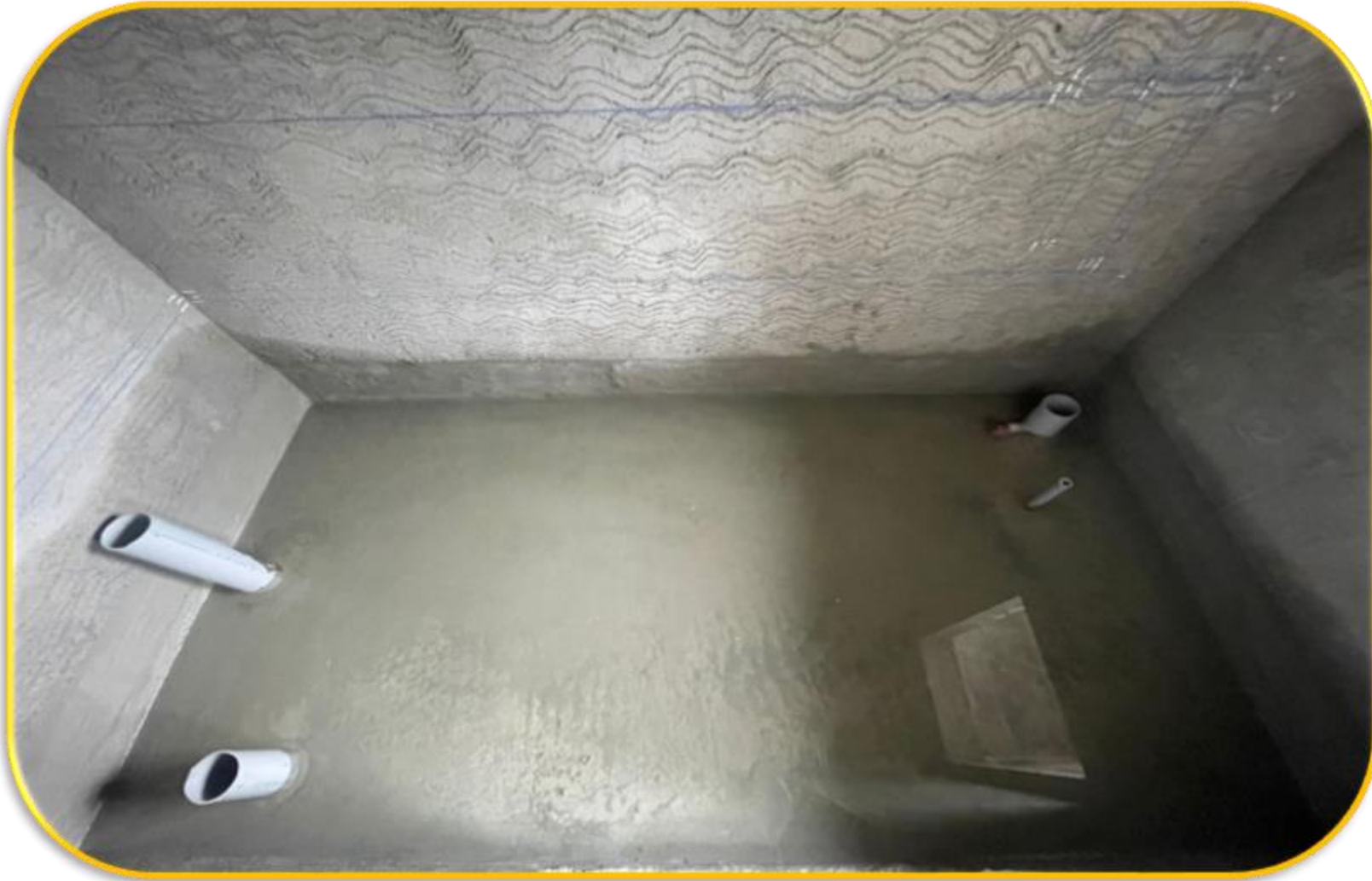
4 th floor toilet water proofing work in progress
