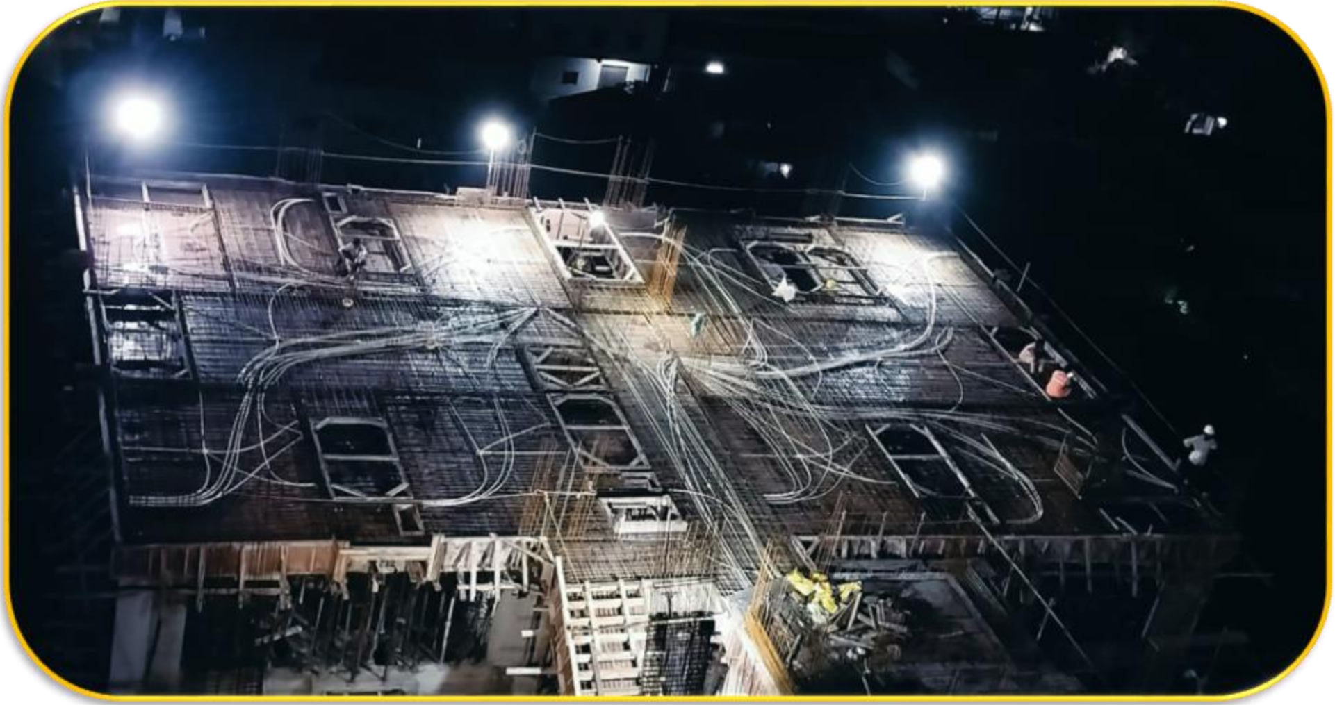
Pour 2 – 11 th Floor roof electrical conduit laying work completed.
