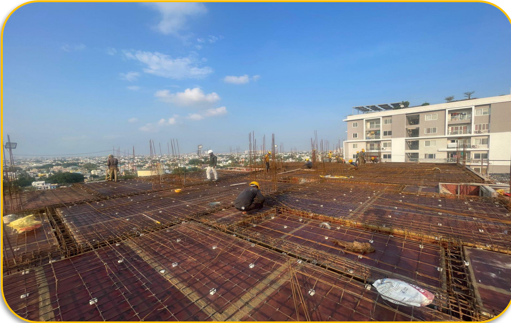
Pour 2 – 10 th Floor roof reinforcement work completed.
