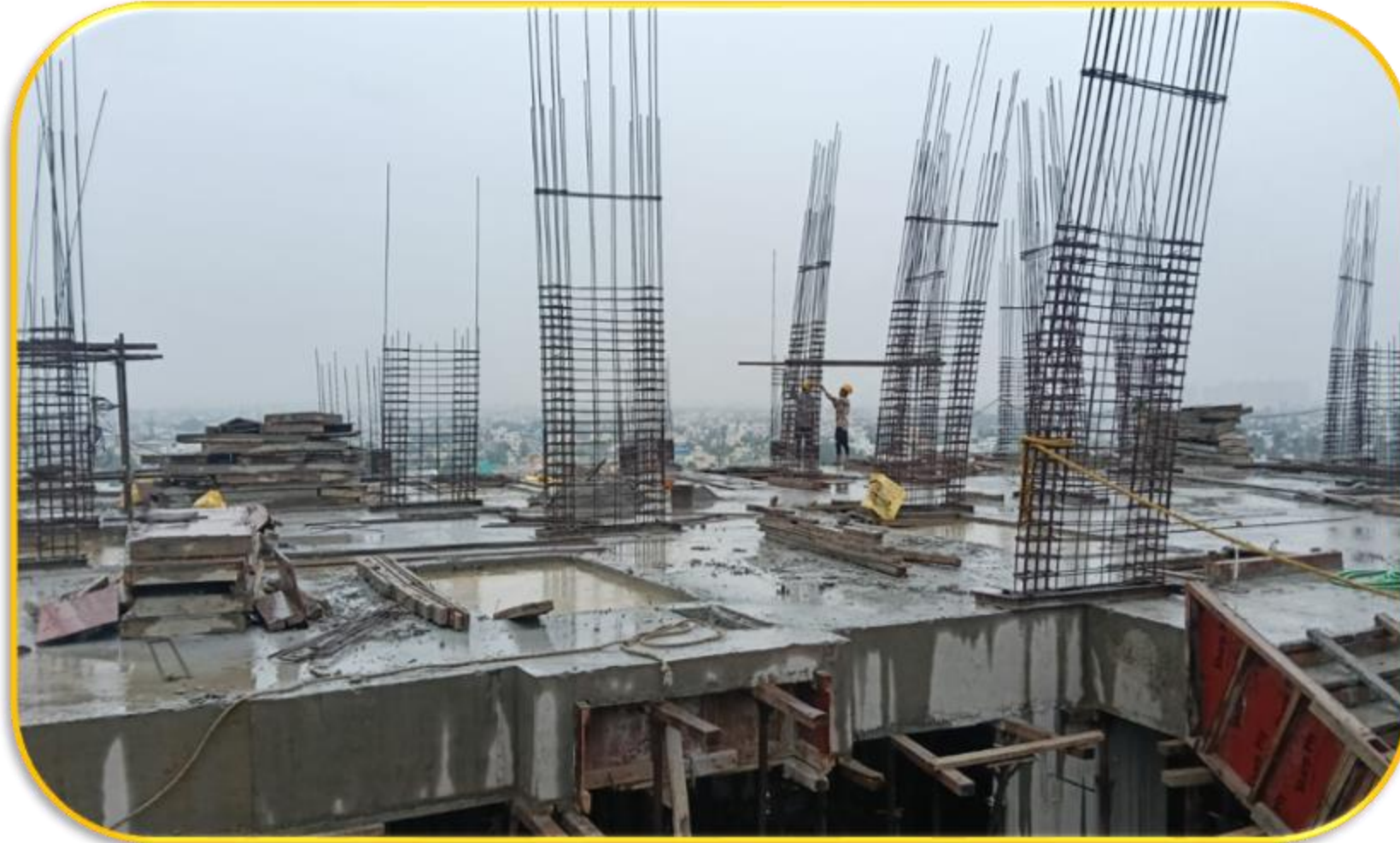
Pore 2 - 12 th floor column reinforcement work in progress
