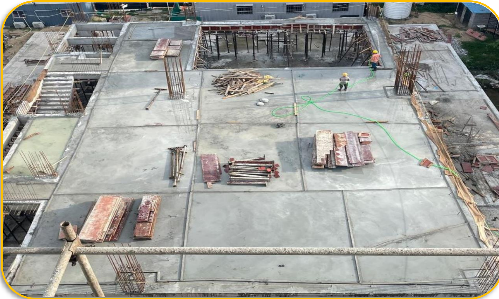
Tower -2 stilt floor roof slab curing work completed.
