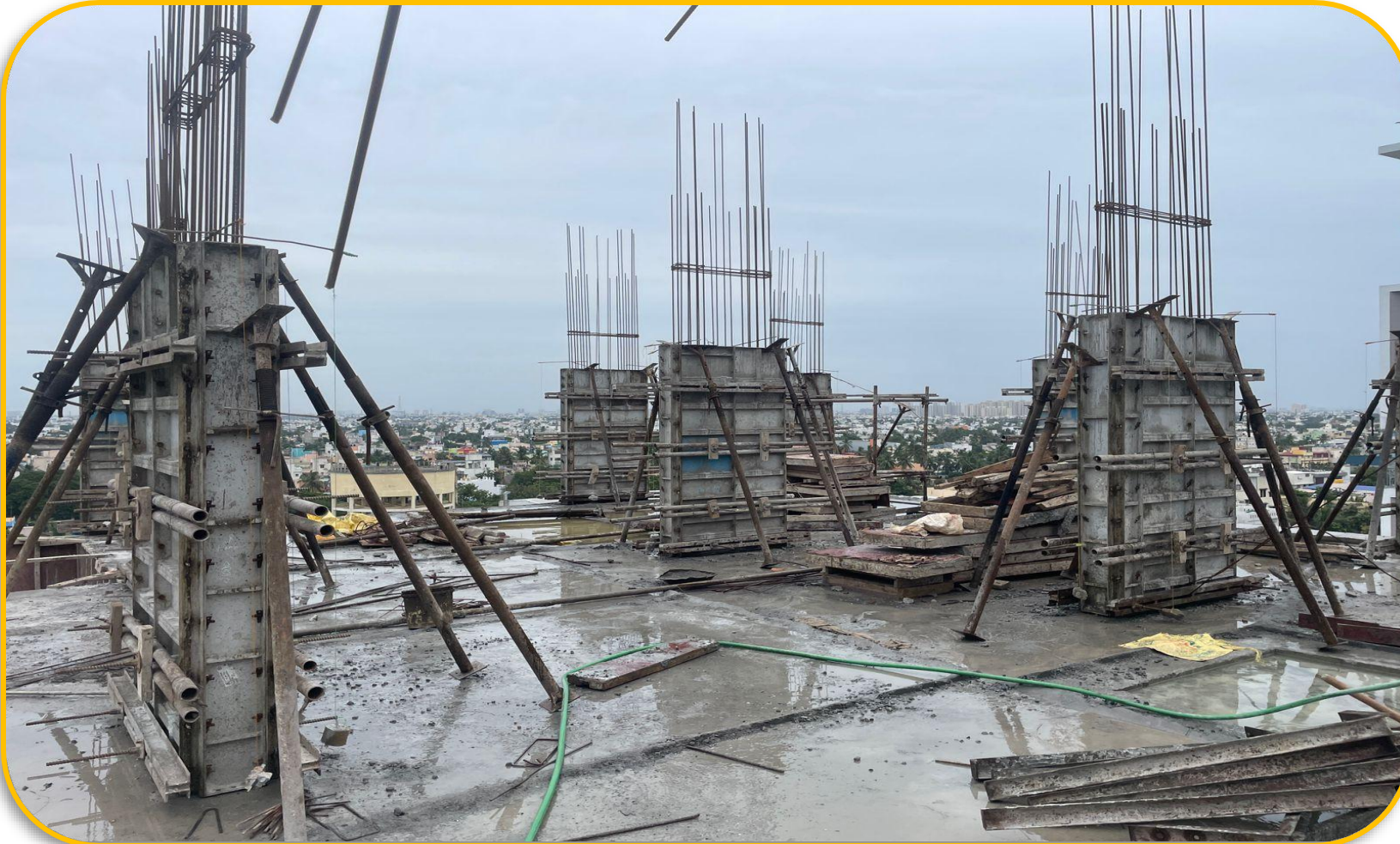
Pour 2 – 10 th Floor column concrete work completed.
