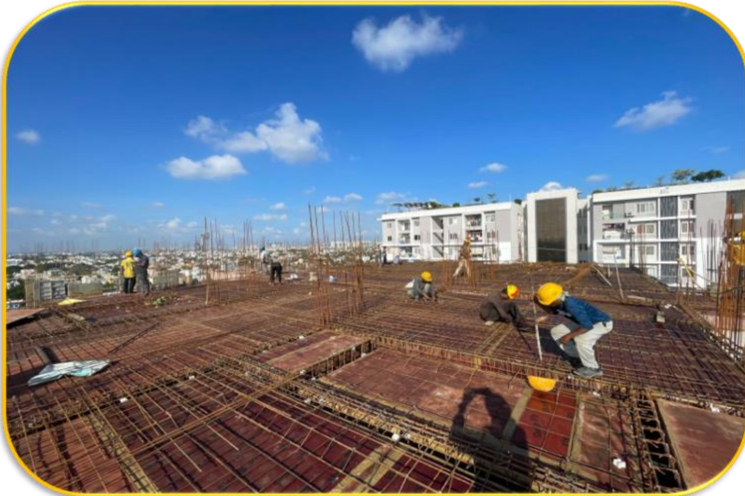
Pour 1 – 11 th Floor roof reinforcement work completed.
