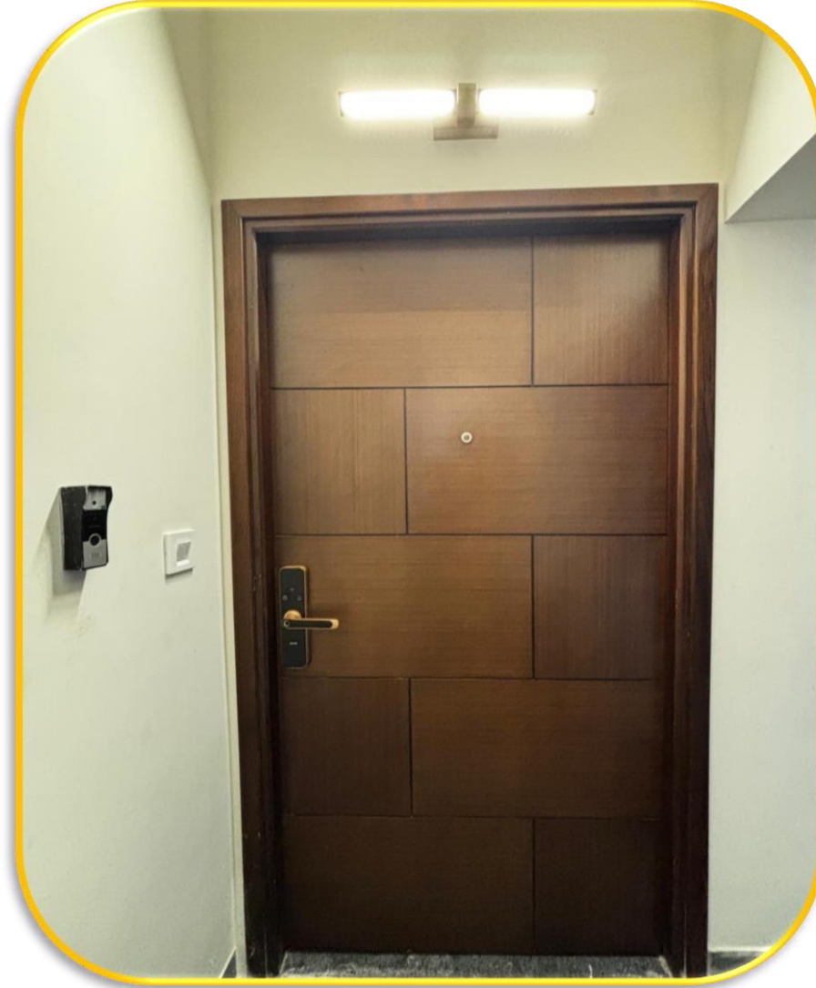
MOCKUP FLAT - MAIN DOOR
