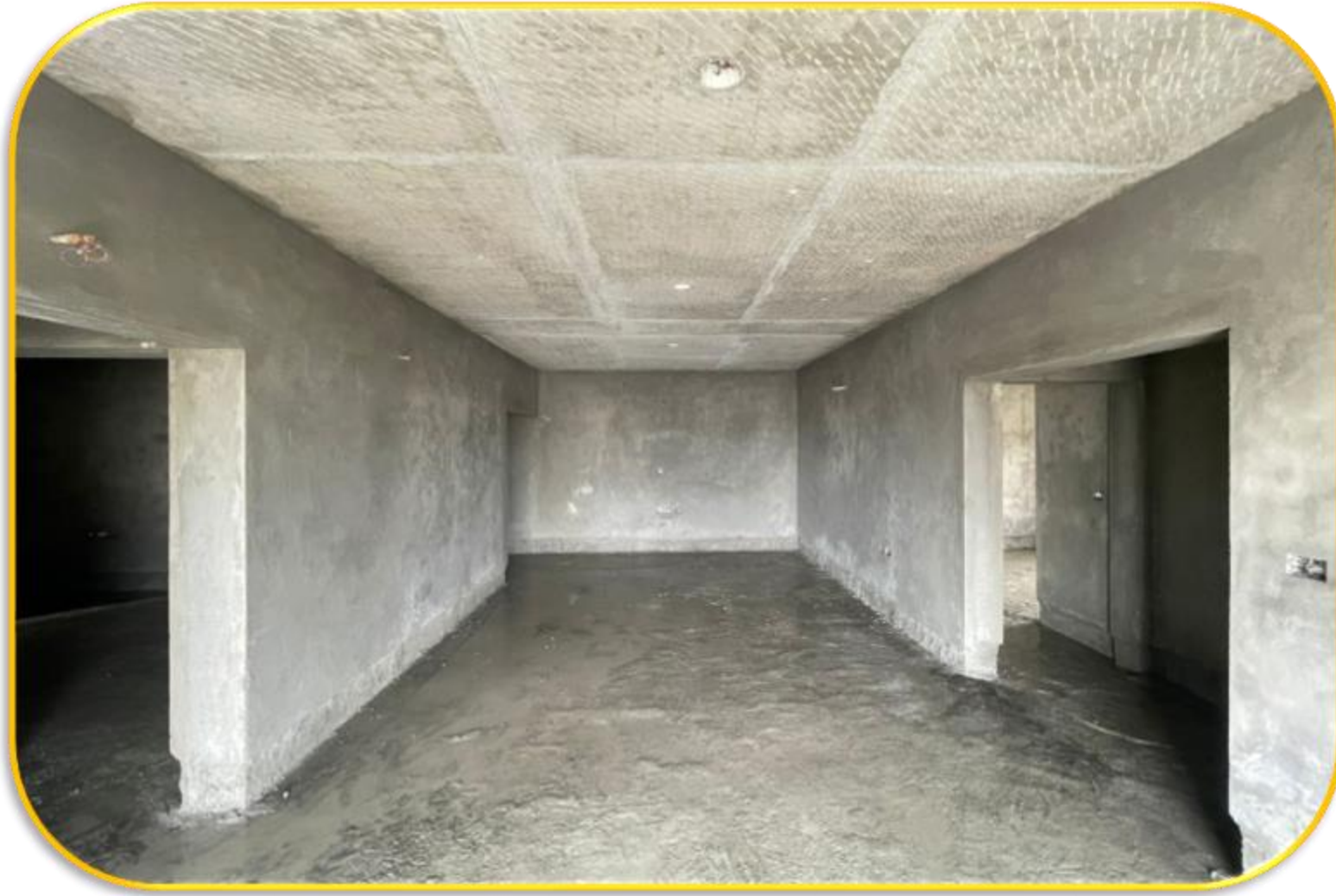
4 th floor inner wall plastering work completed
