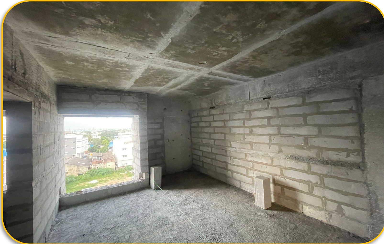
6 th Floor block work completed.
