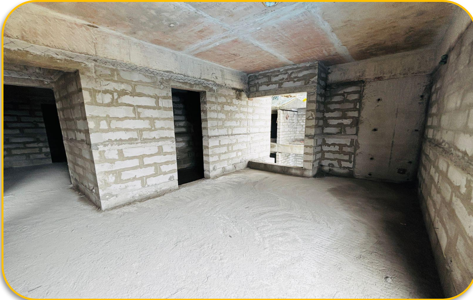
8 th Floor block work in progress.
