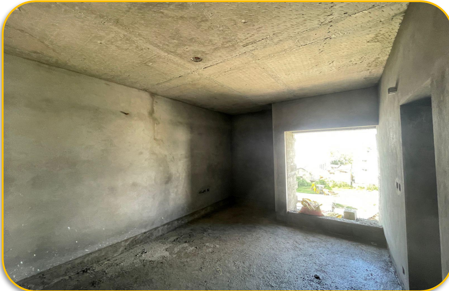
5 th Floor plastering work in progress.
