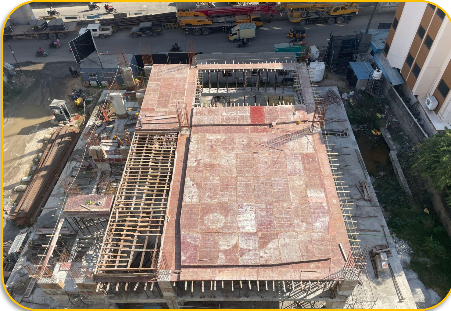
Tower 2 1 st floor roof shuttering work in progress
