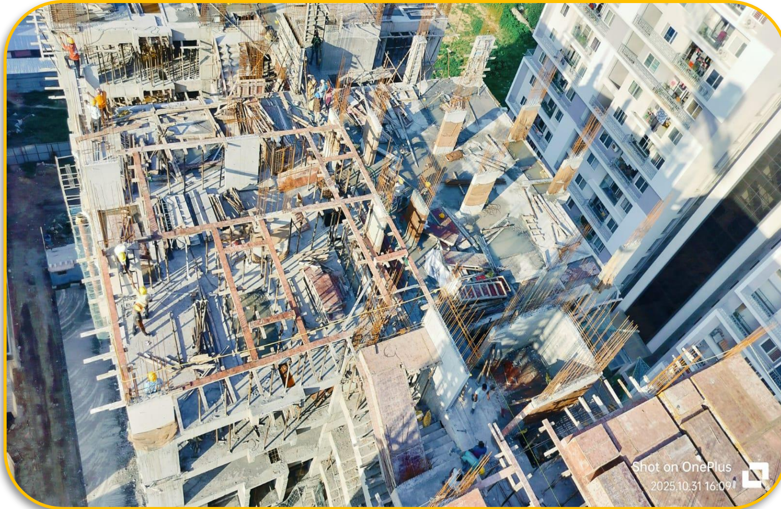
North Side View
