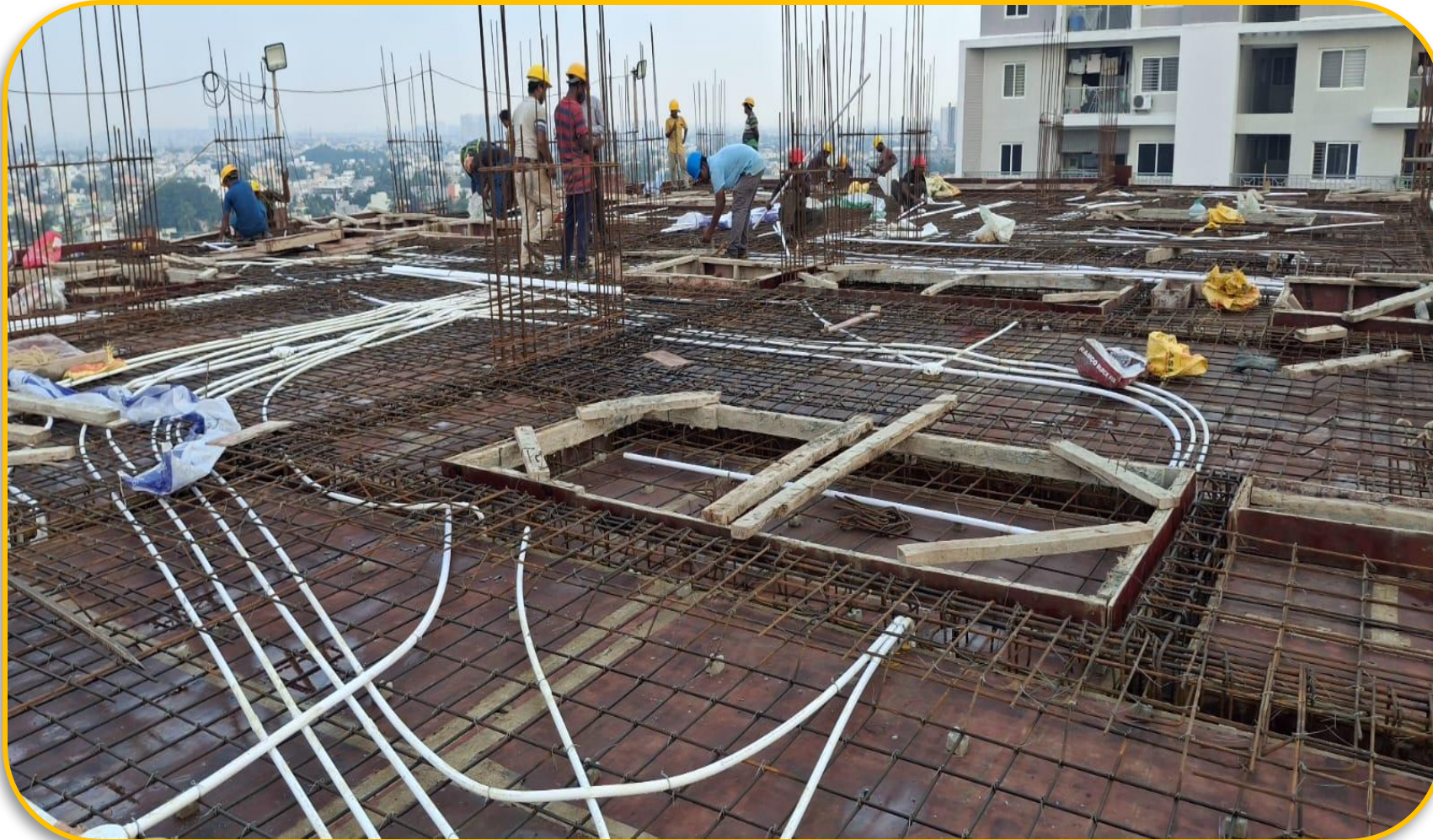
Pour 2 – 10 th Floor roof electrical conduit laying work completed.
