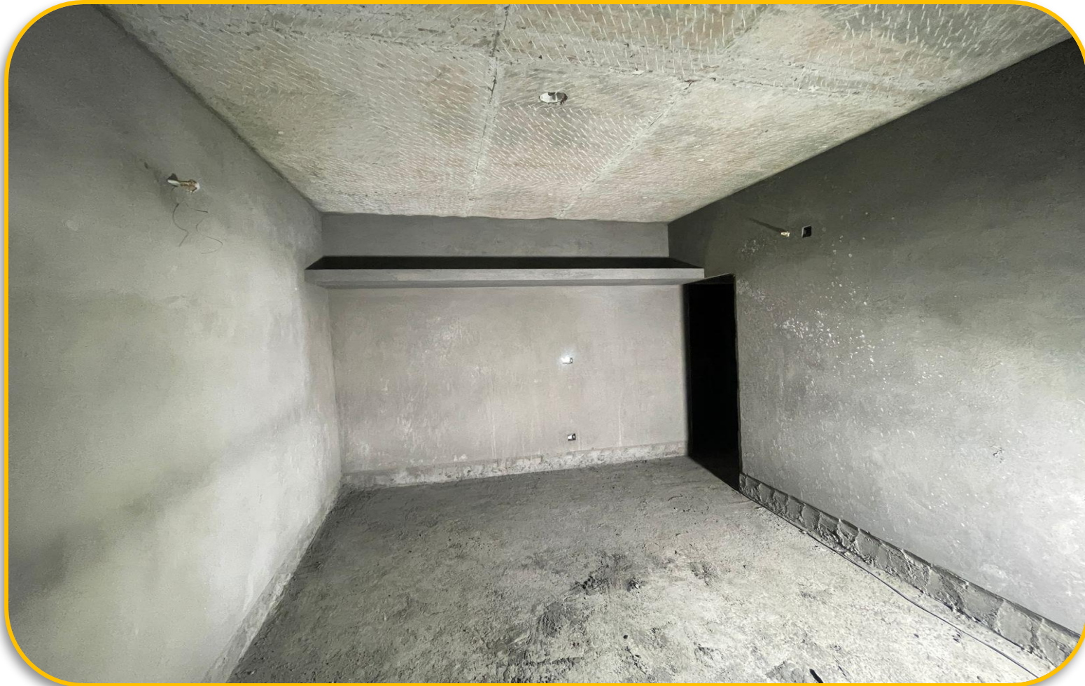
3 rd floor inner wall plastering work completed.
