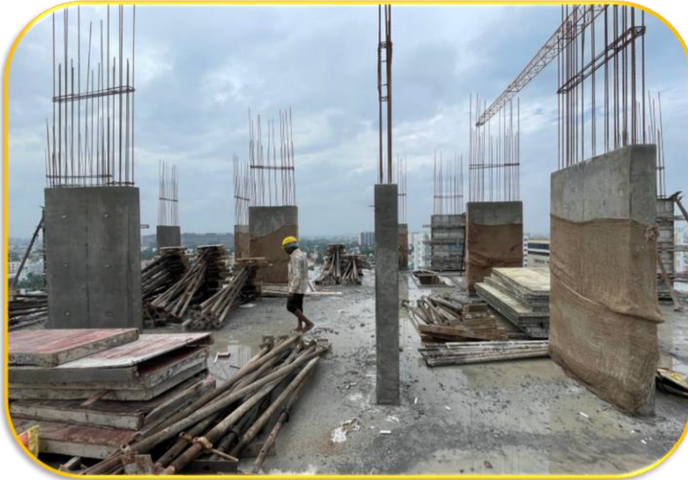
Pour 1 – 12 th floor column concrete work in progress
