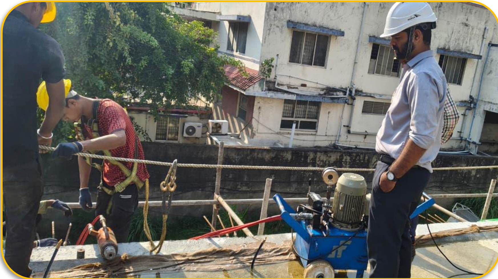
Tower -2 stilt floor roof PT strand stressing work completed.
