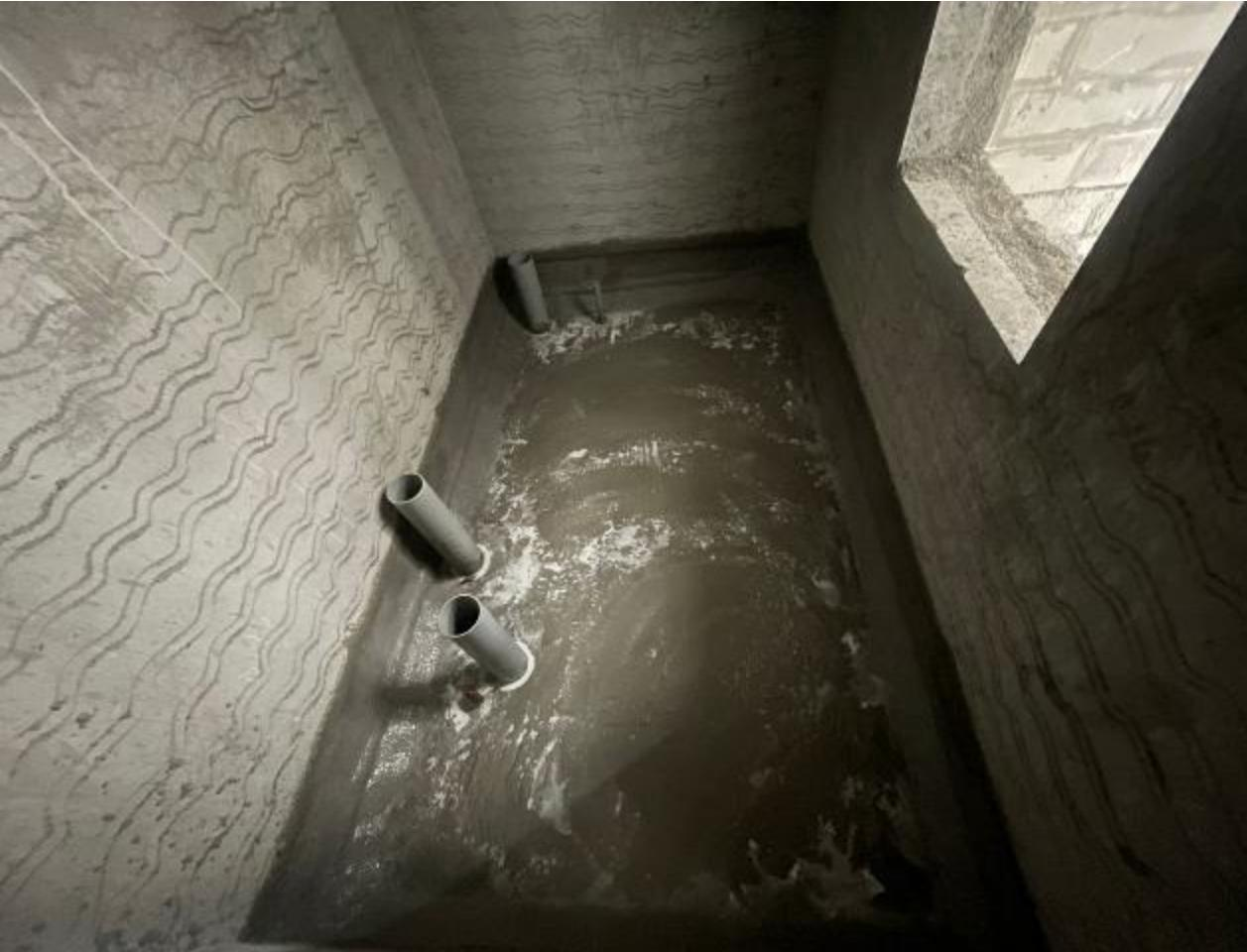
**6<sup>th</sup> FLOOR TOILET AND BALCONY SUNKEN FILLING WORK IN PROGRESS**
