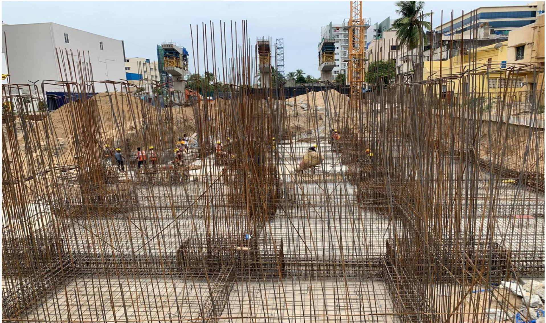
Pour 1 – Part 1 raft slab reinforcement work in Progress.
