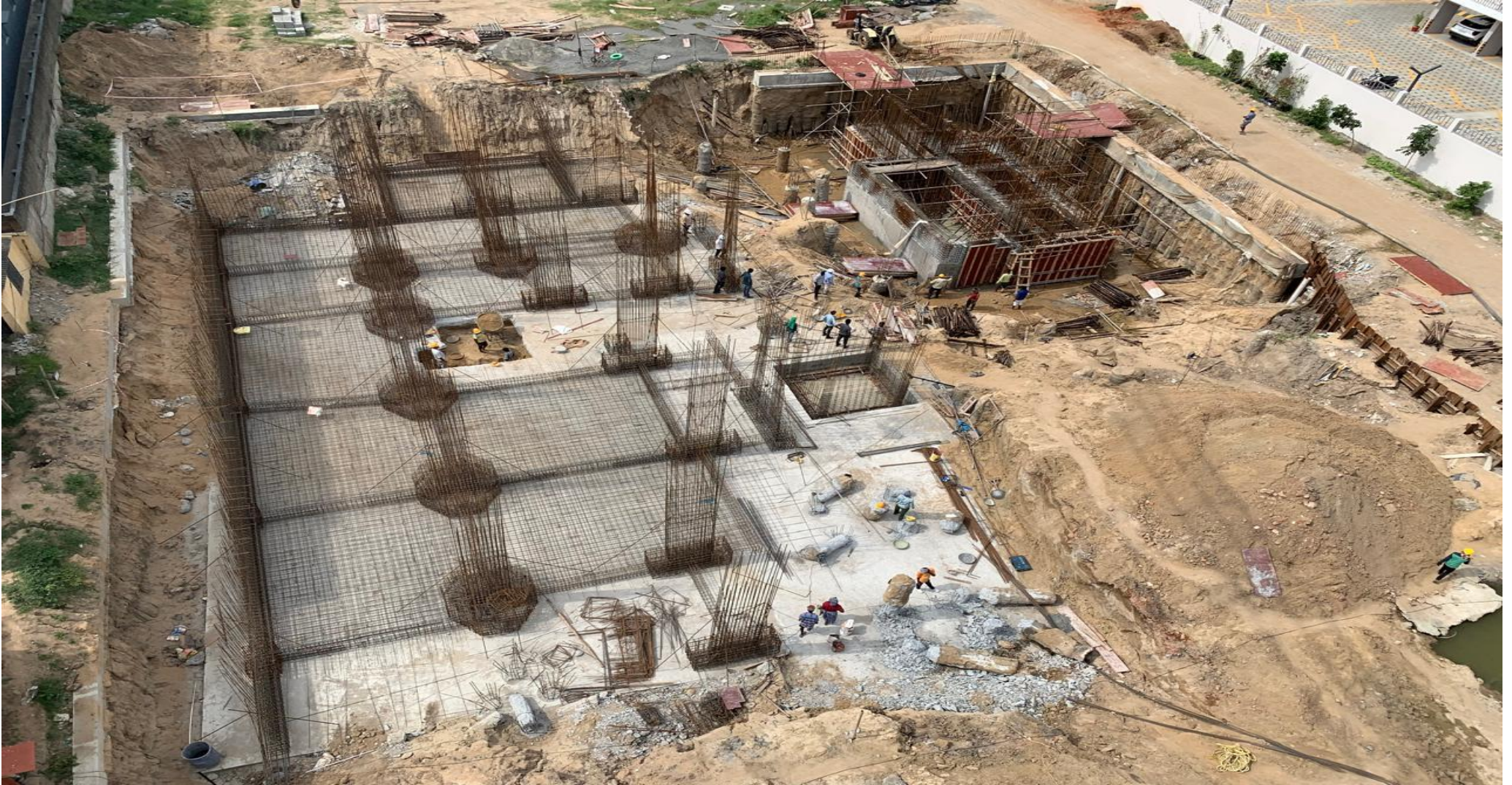
North Side View
