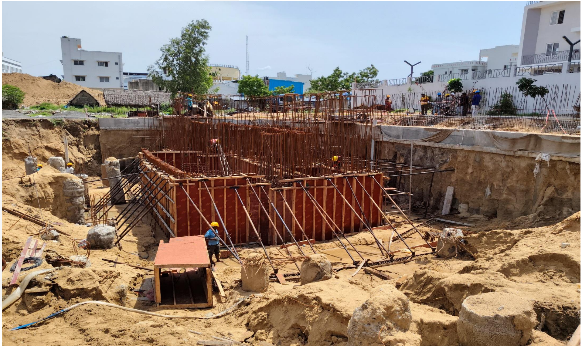
STP Wall 1 st lift shuttering work completed.
