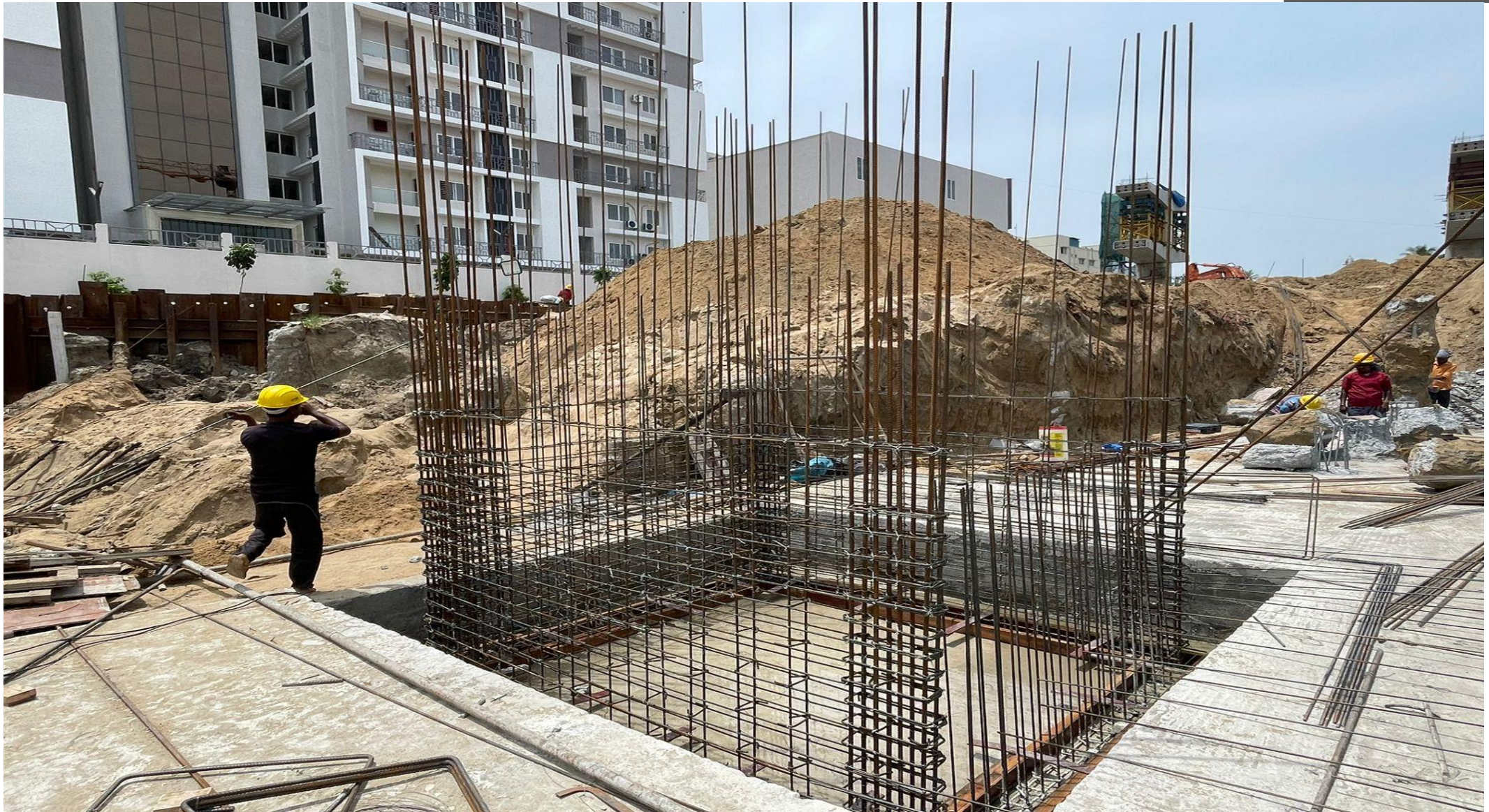
Lift wall reinforcement work completed.
