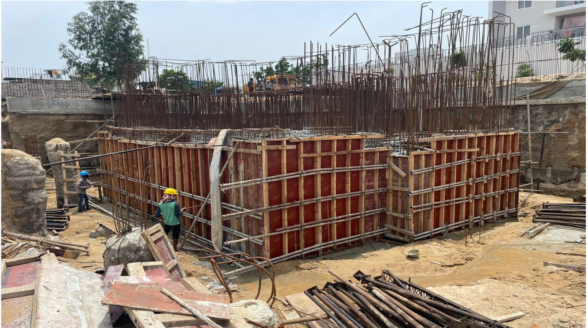
STP 1 st lift Wall de-shuttering works in progress.
