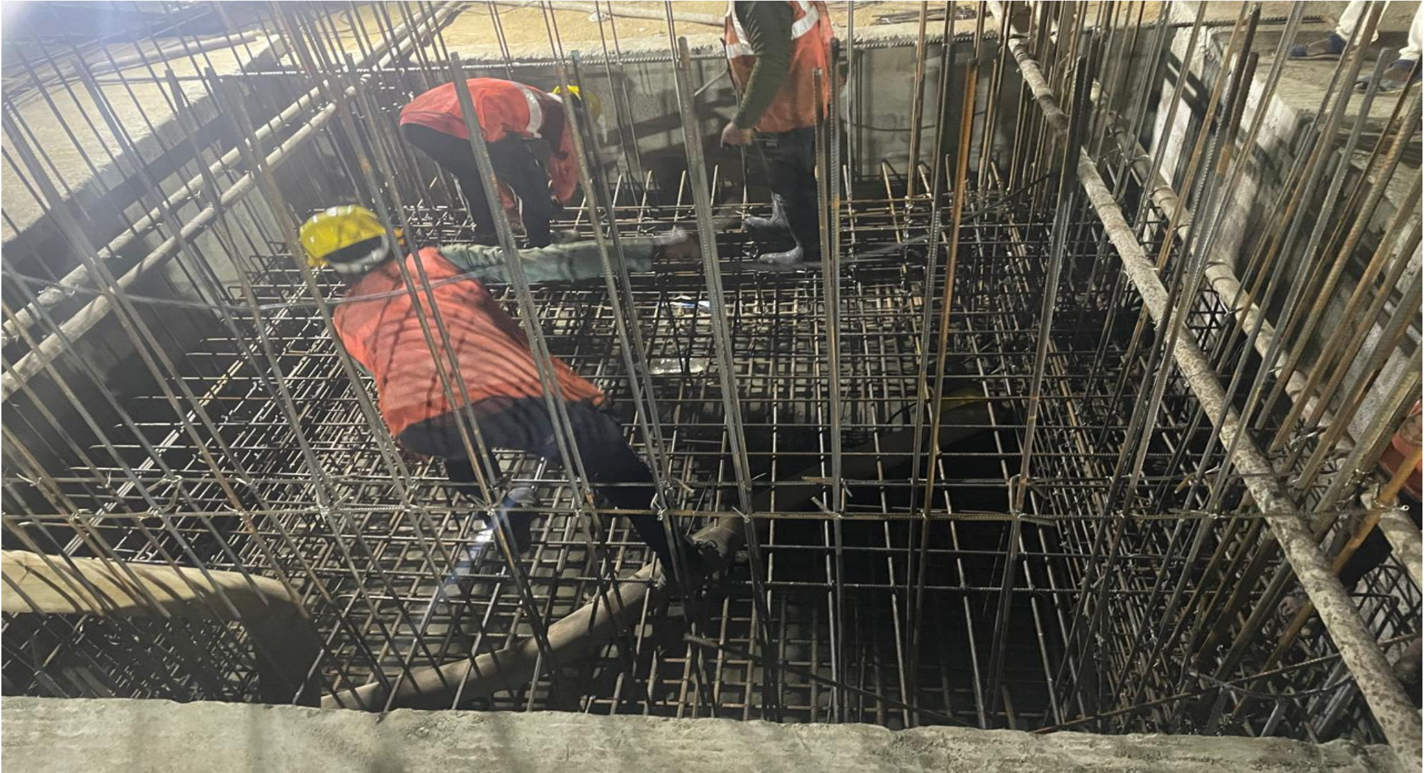
Lift pit raft concrete completed.
