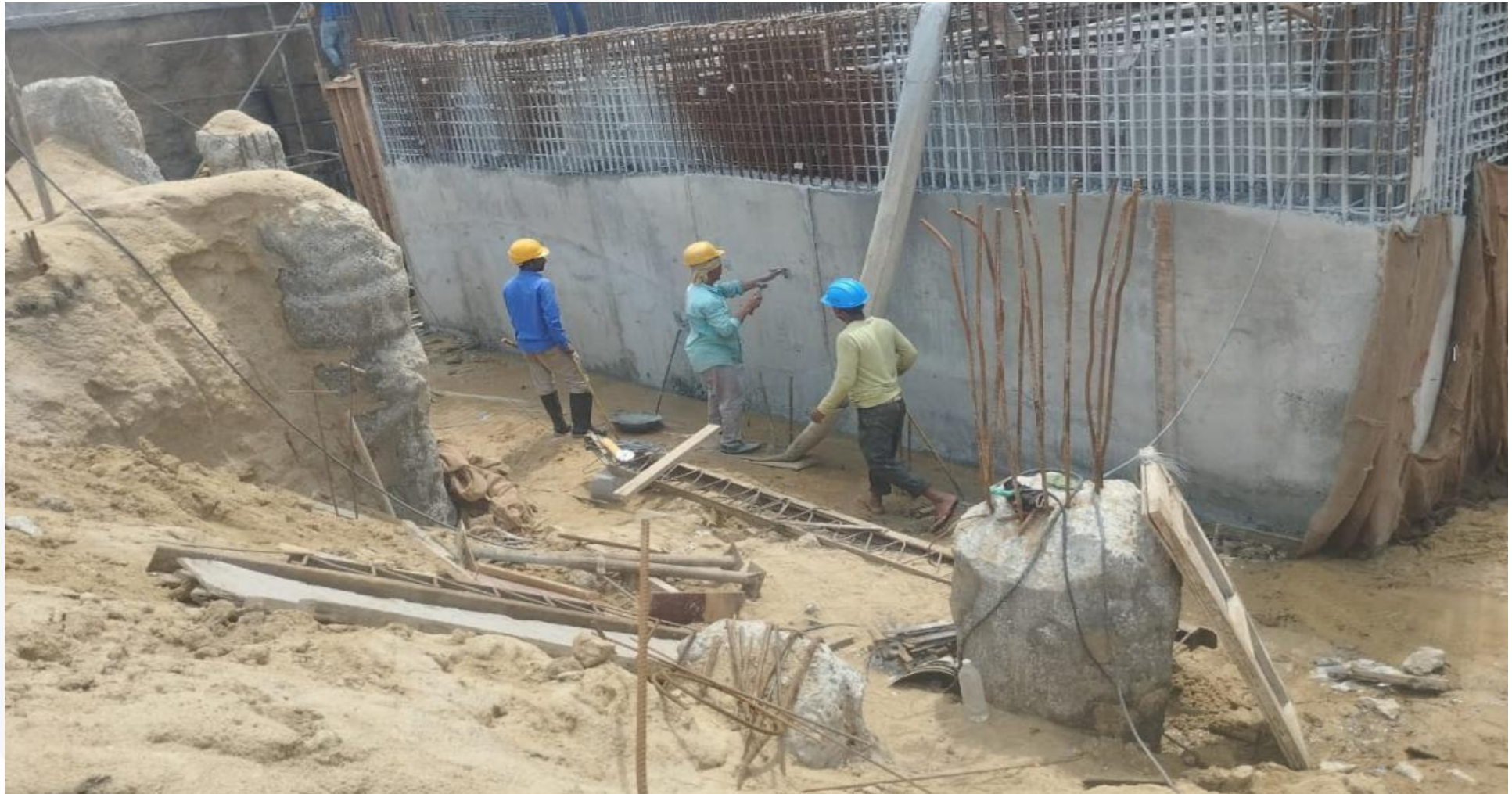
STP 1 st lift Wall Water proofing preliminary works in progress.
