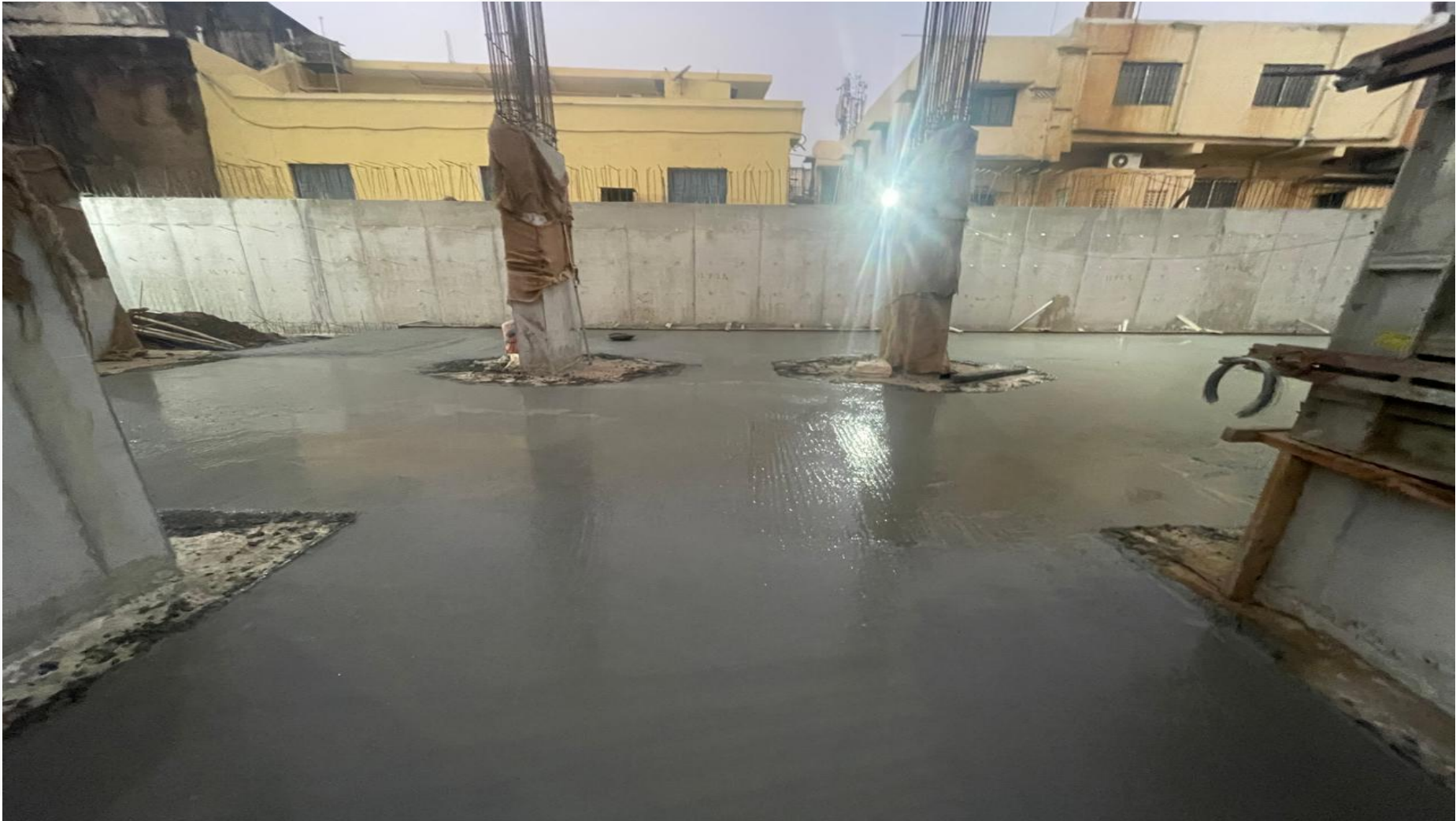
Basement pour-1 grade slab concreting work completed.
