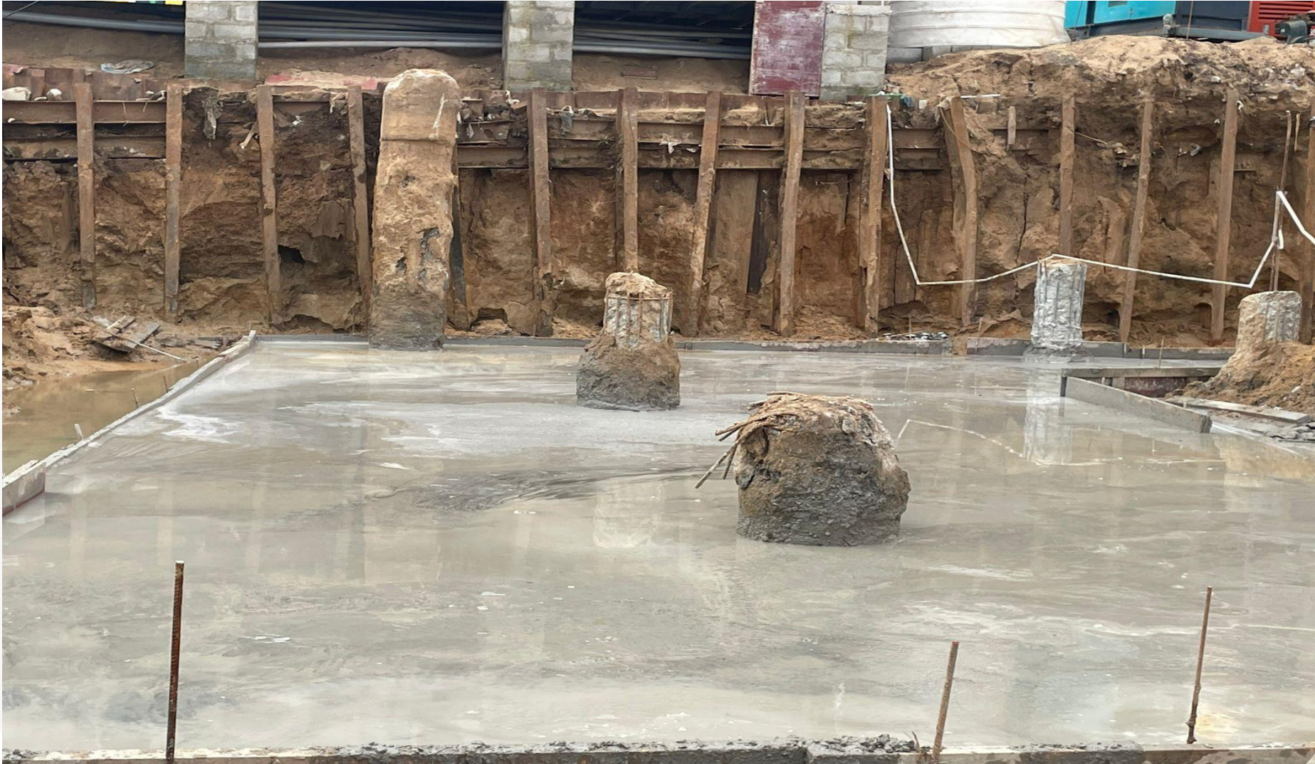
Pour-3 PCC concreting work completed.
