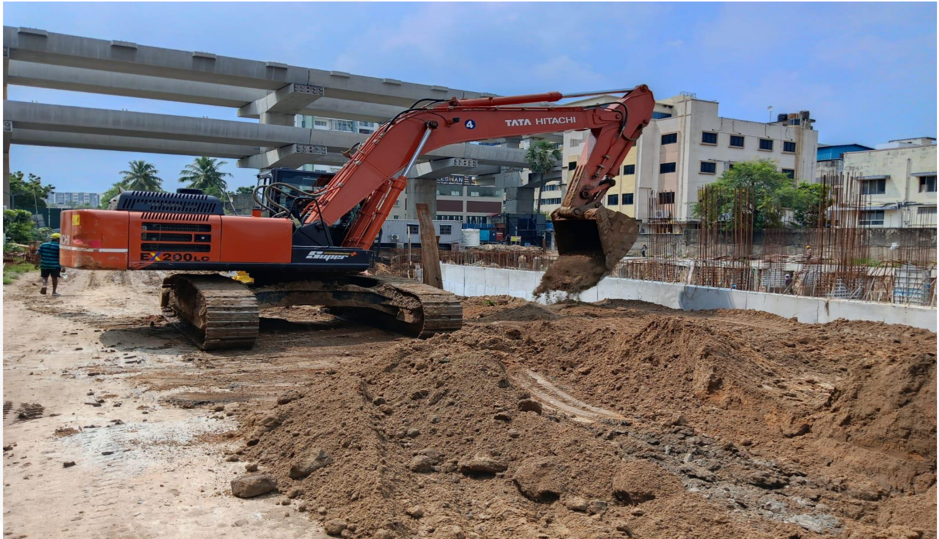
East side soil backfilling work in progress.
