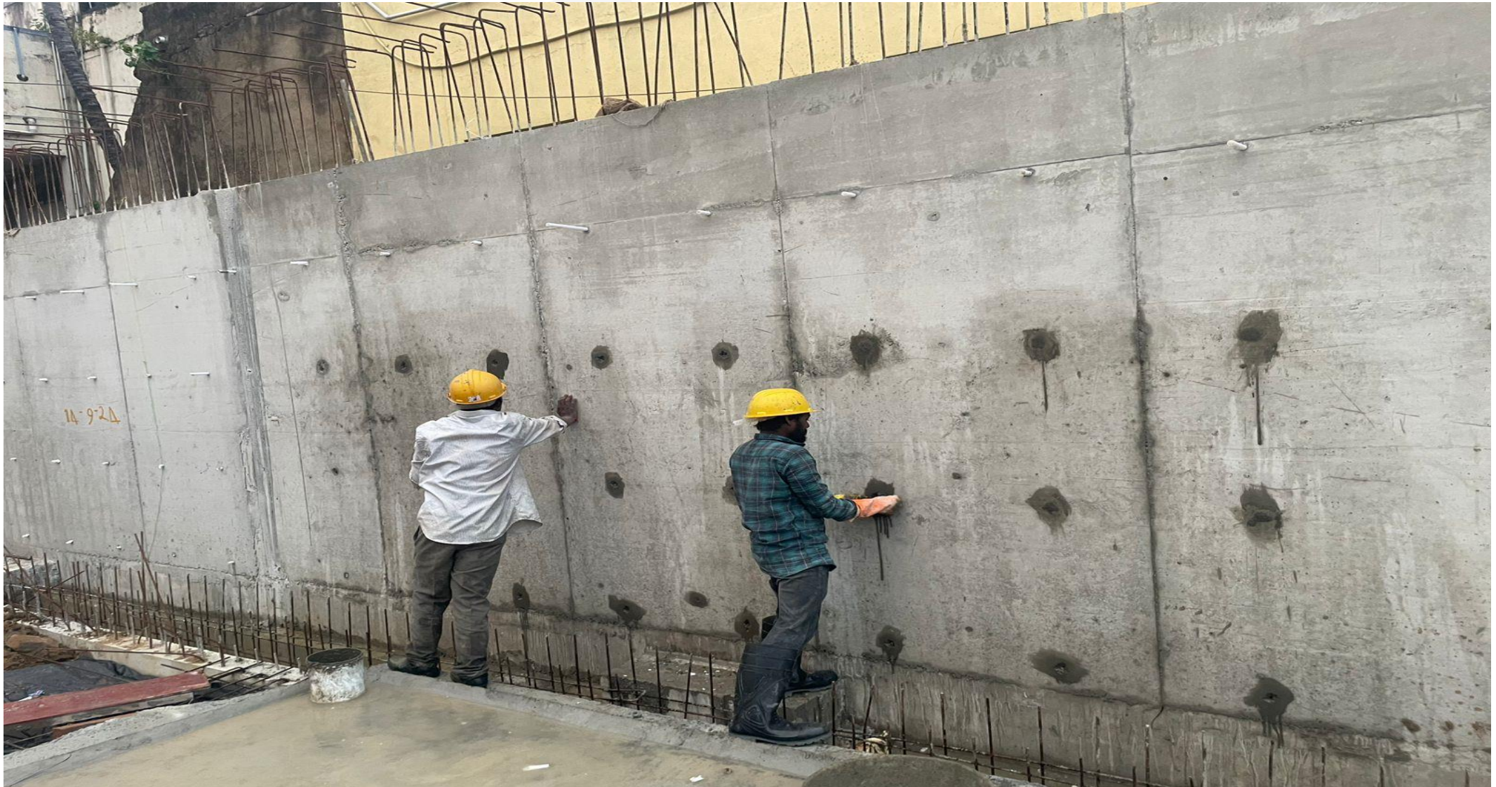
West-side retaining wall waterproofing work in progress.
