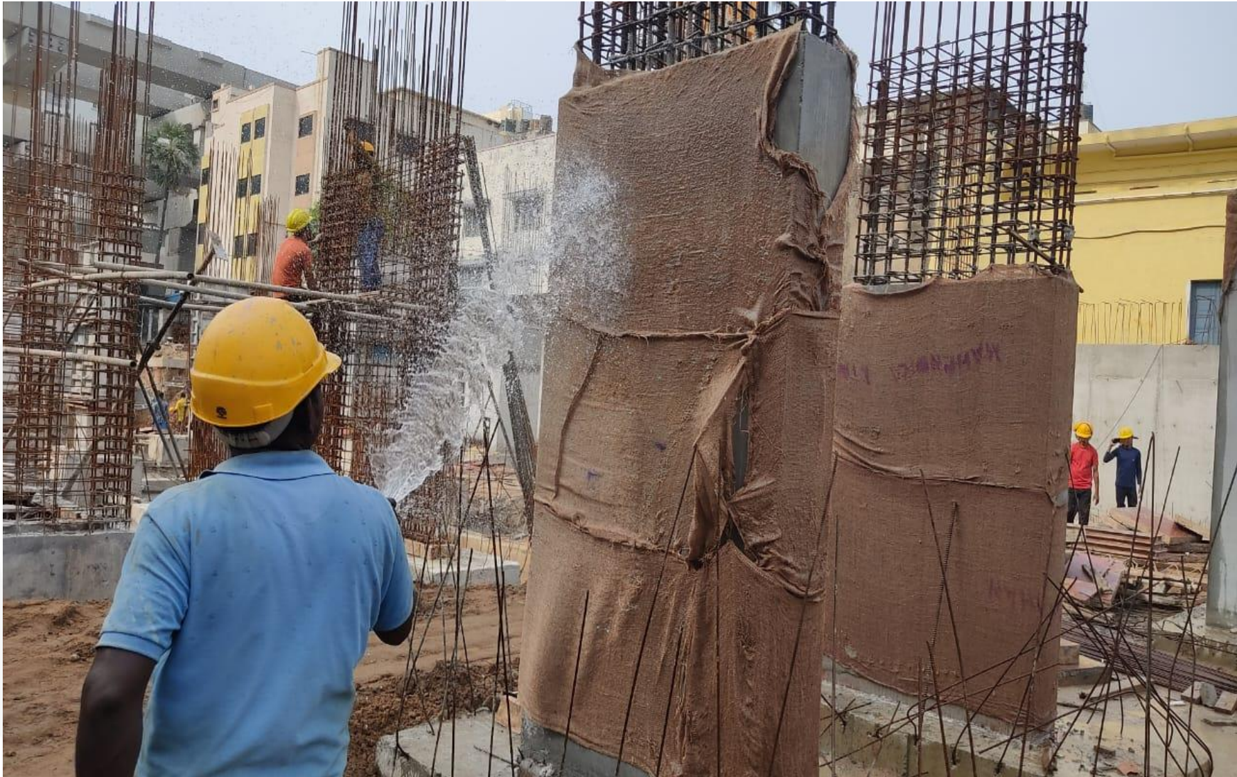
Pour-1 column curing work in progress.
