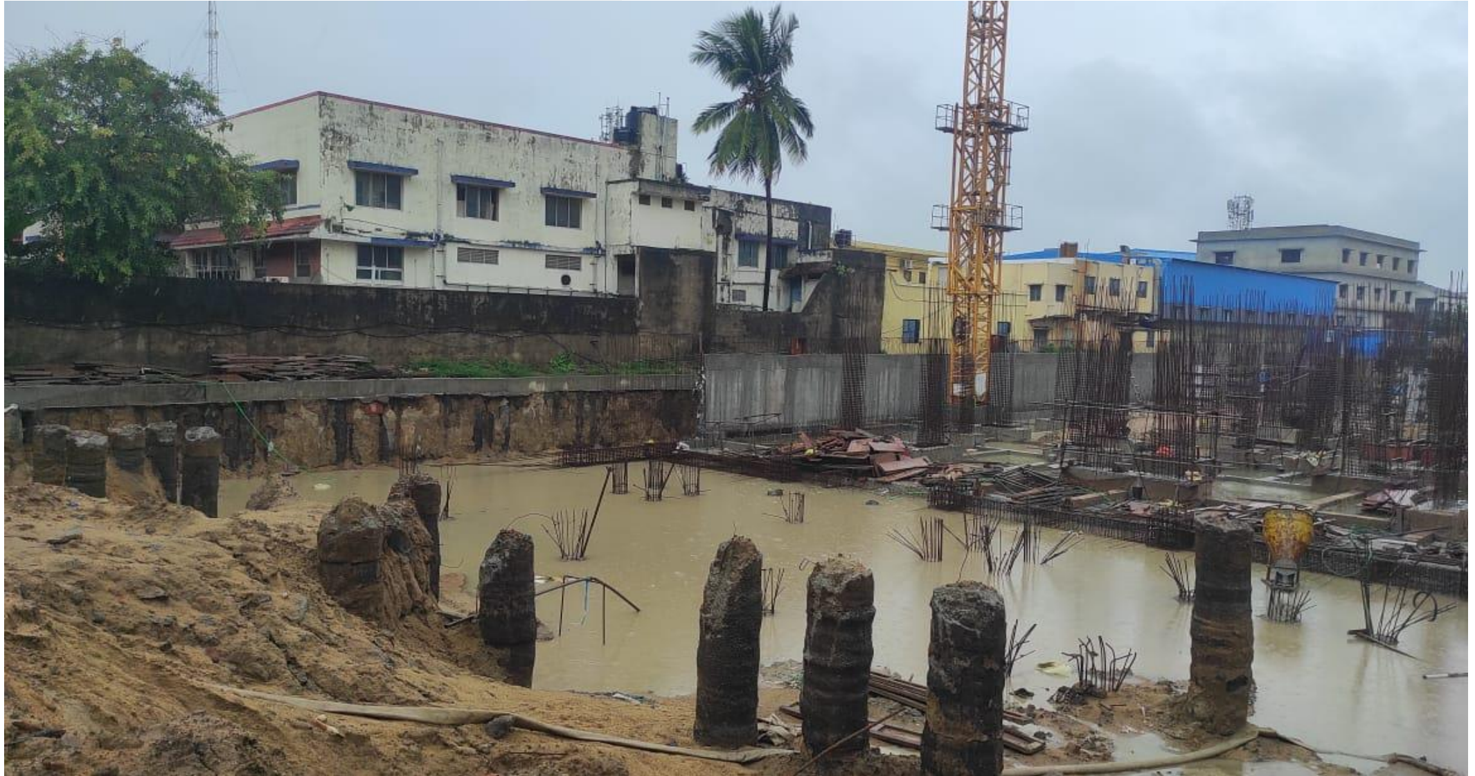
Dewatering work in progress.
