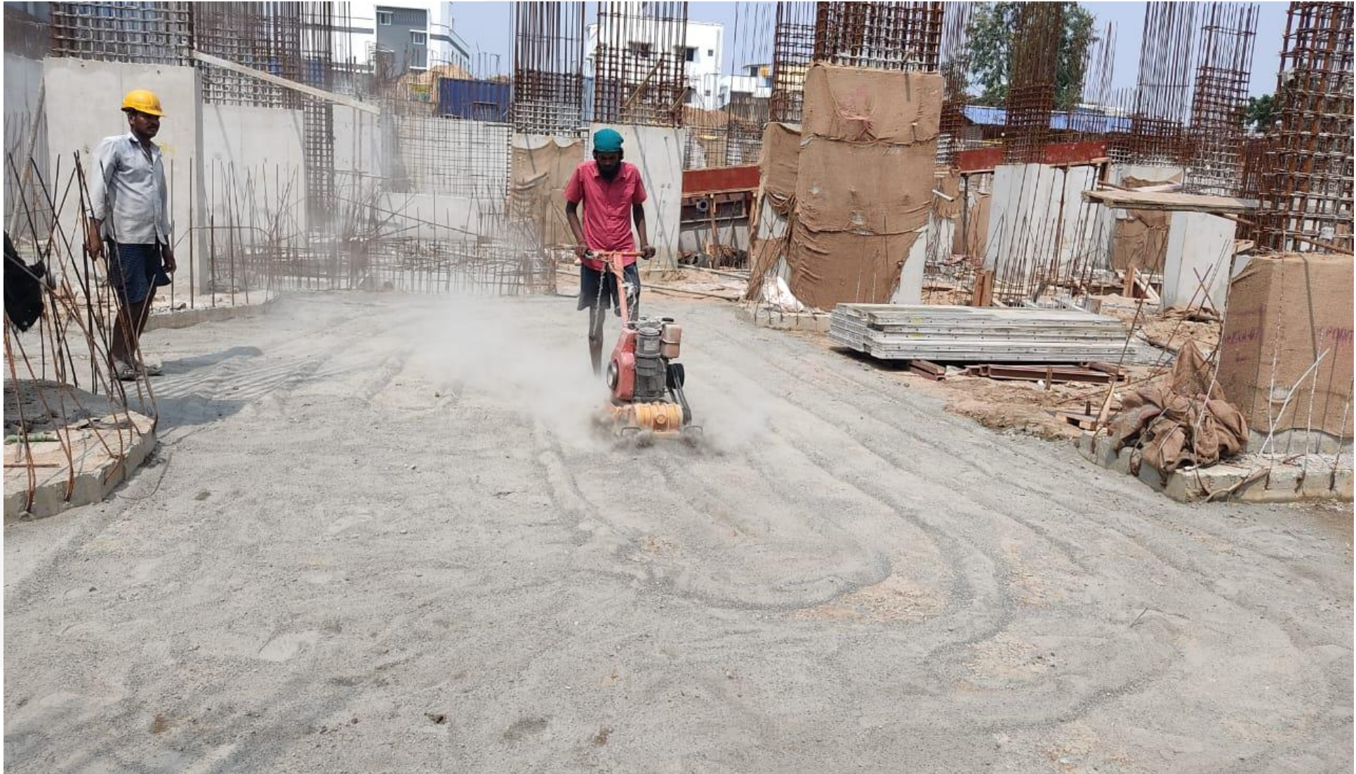
Basement pour-1 soil compaction work completed.
