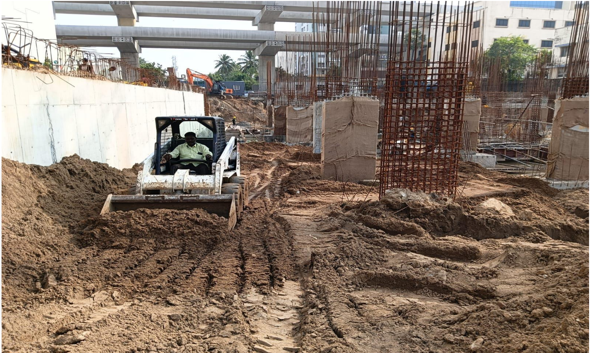
Basement Pour-2 remaining area soil backfilling work in progress.
