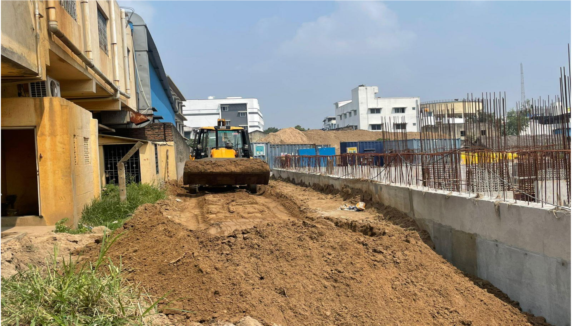
West side outer soil backfilling work in progress.
