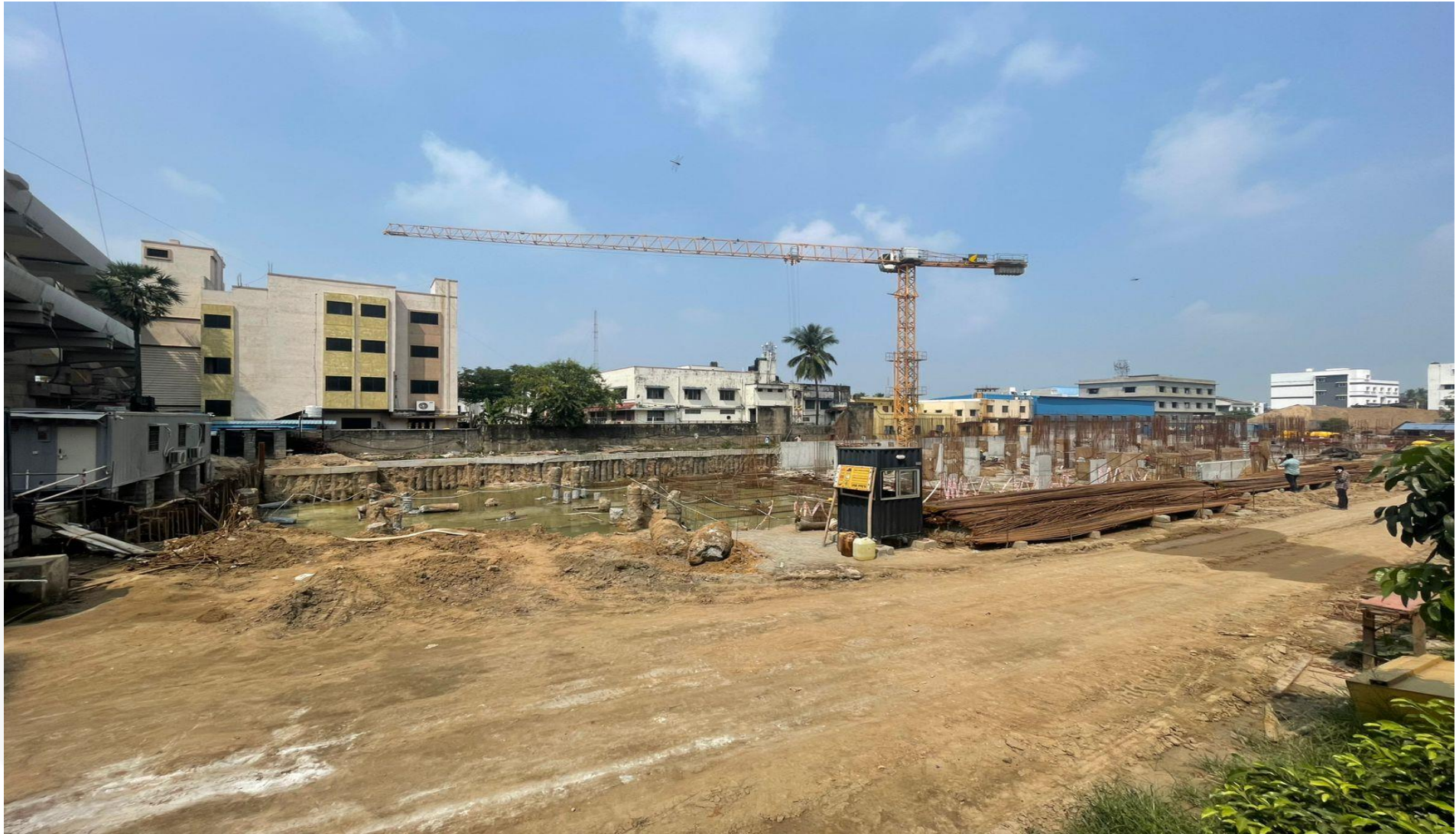
South East corner view.
