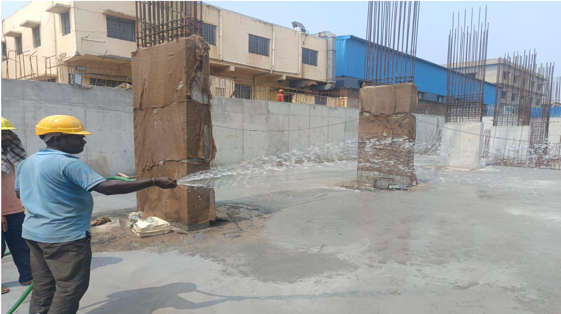
Basement pour-1 grade slab curing work in progress.
