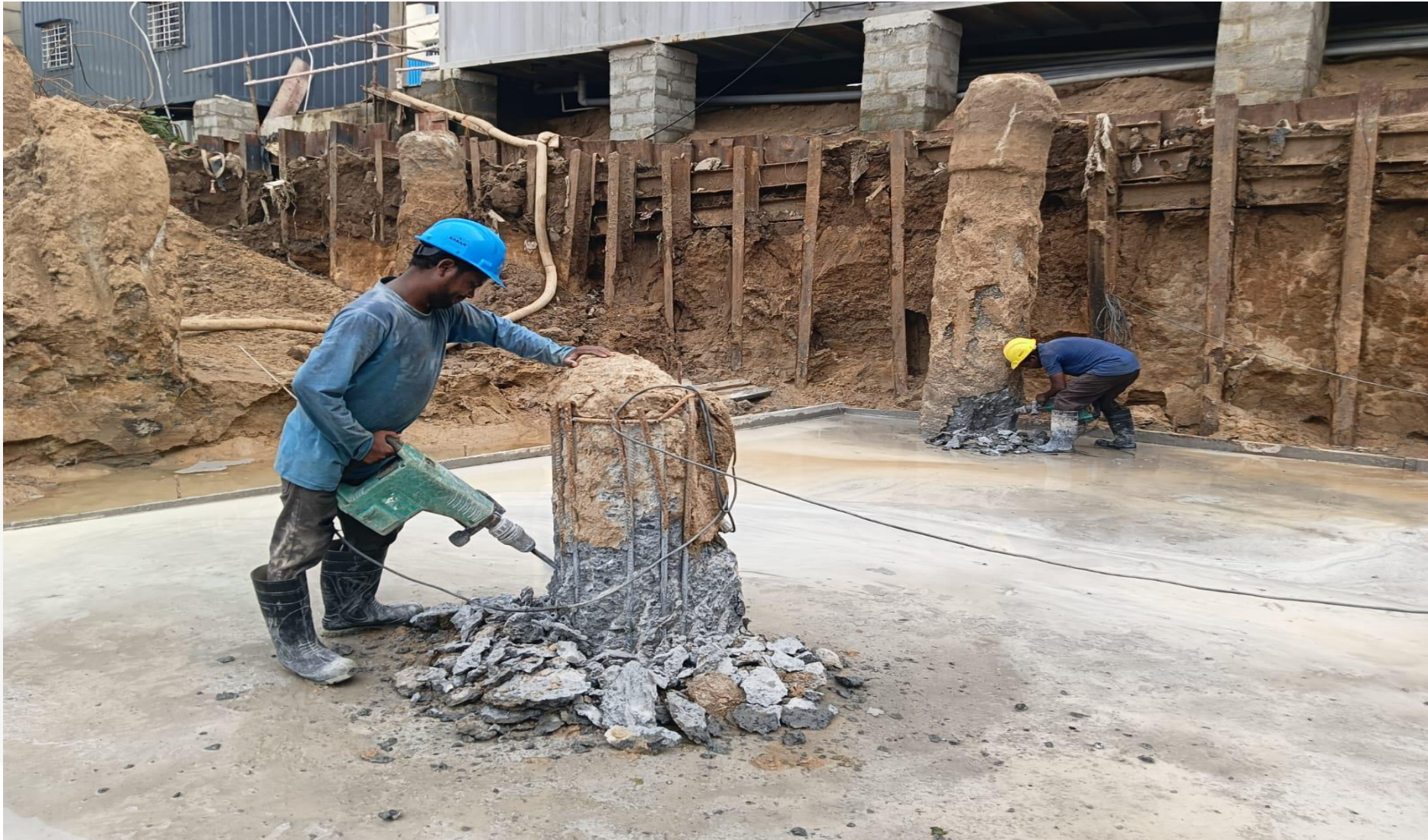
Pour-3 pile cap head chipping work in progress.
