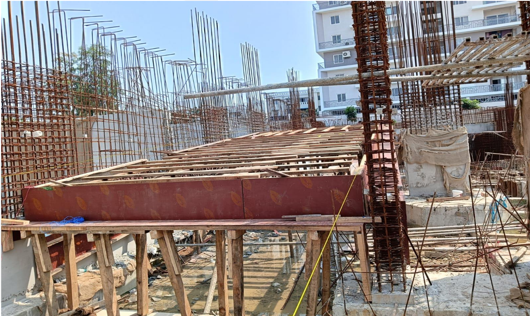
Ramp-1 slab shuttering work in progress.
