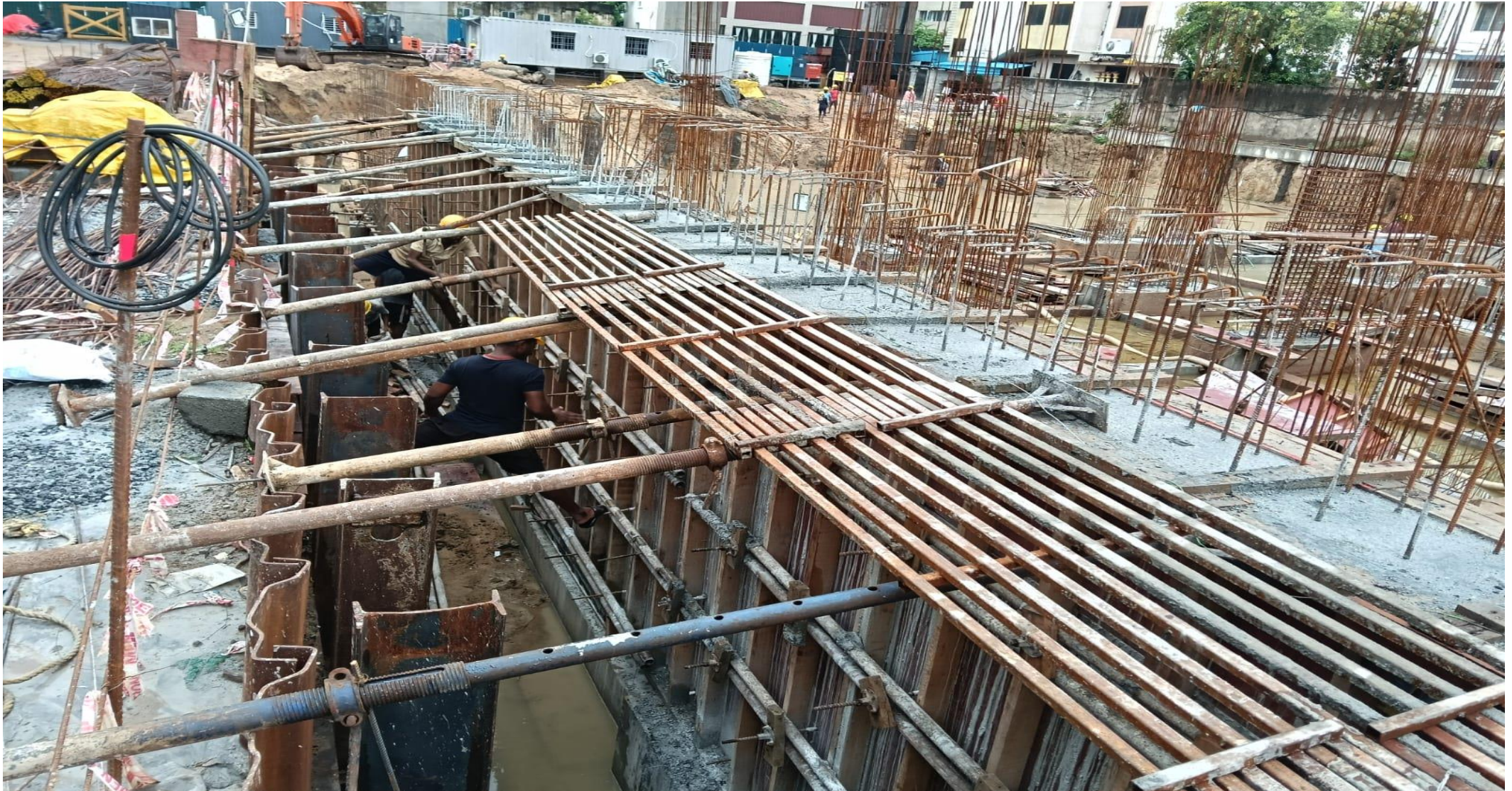
East side retaining wall concrete work completed.
