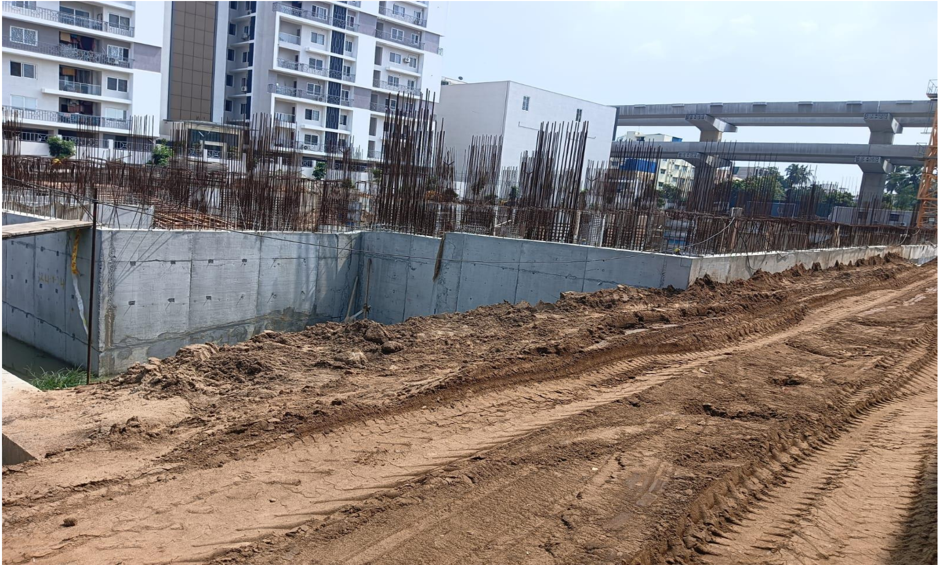
North West corner view.
