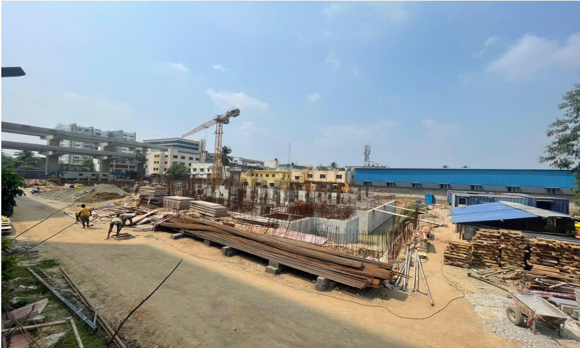
North east corner view.
