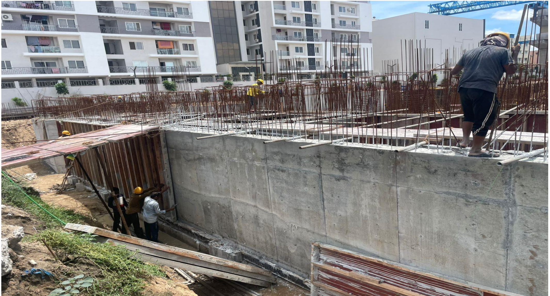
UG sump wall Concrete work completed.
