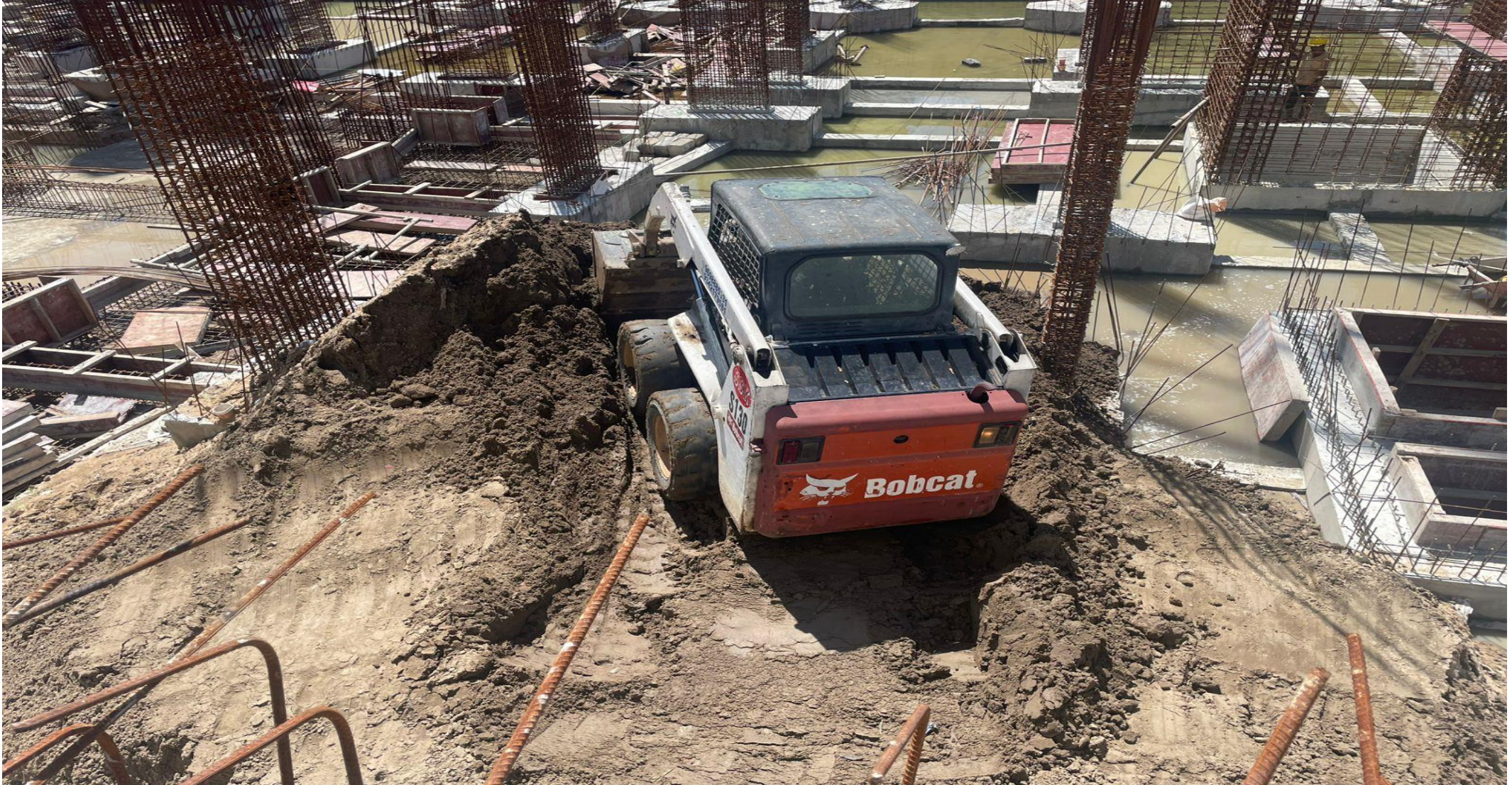
T-01 Basement floor soil backfilling work in progress.
