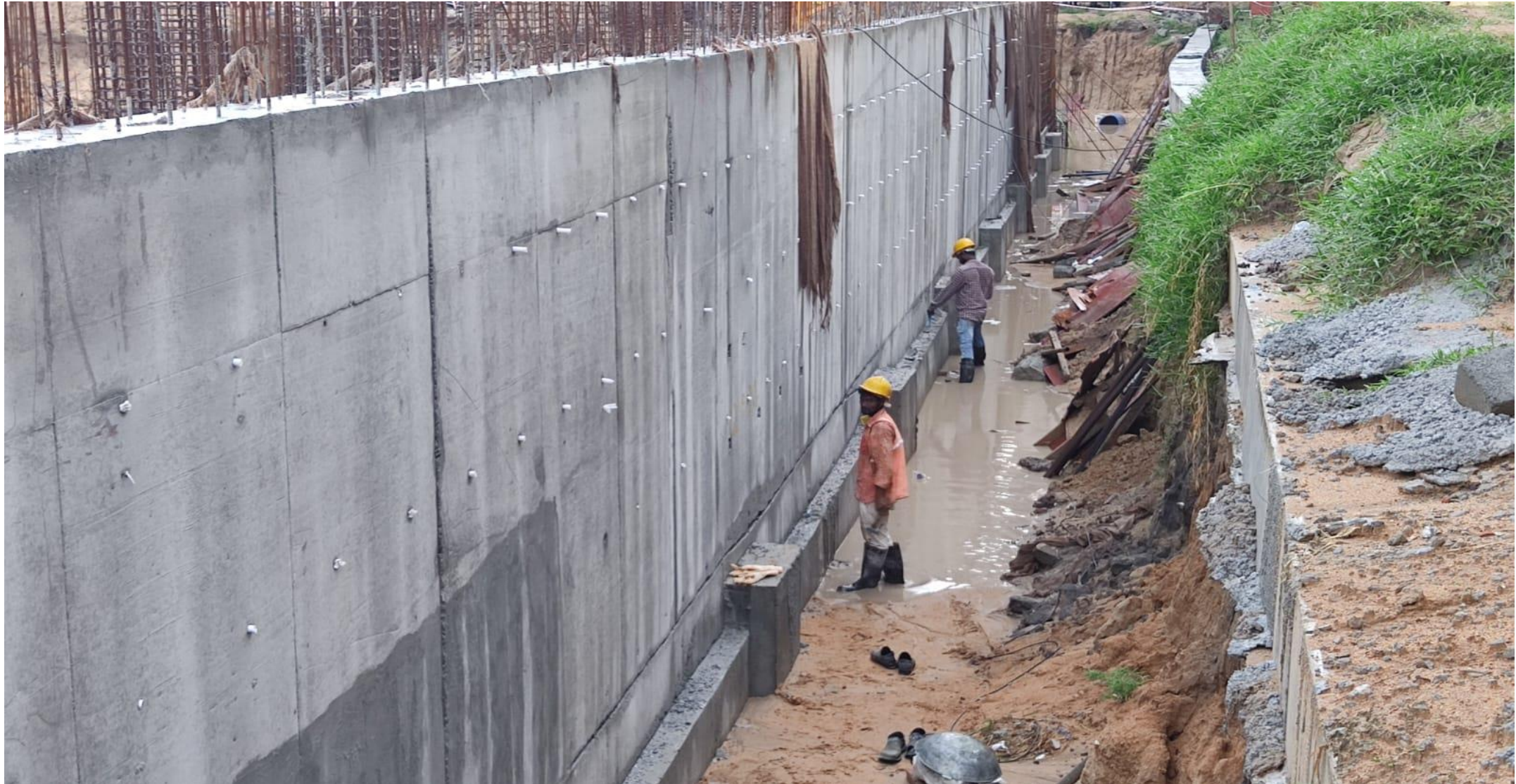
West side retaining Wall water proofing work in progress.
