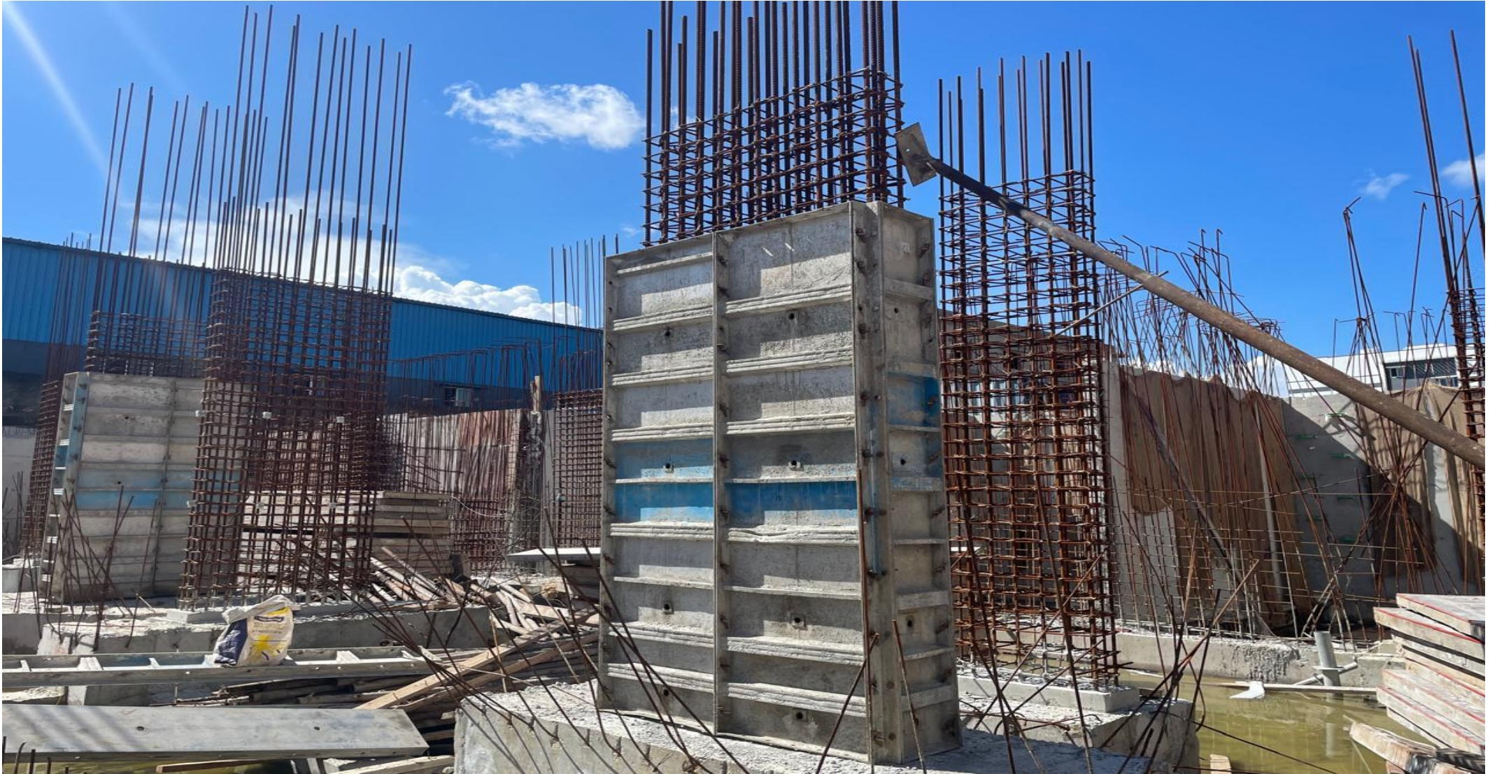
T-1 Column Shuttering work in progress.
