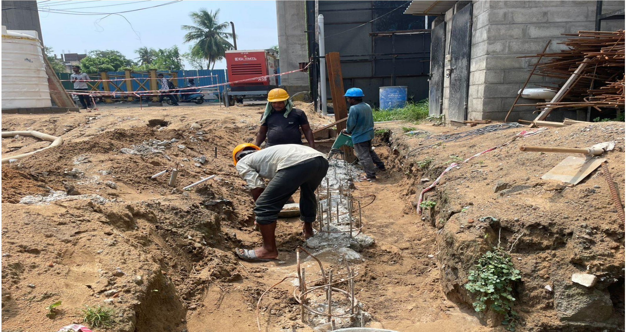
West side contiguous pile chipping work in progress.
