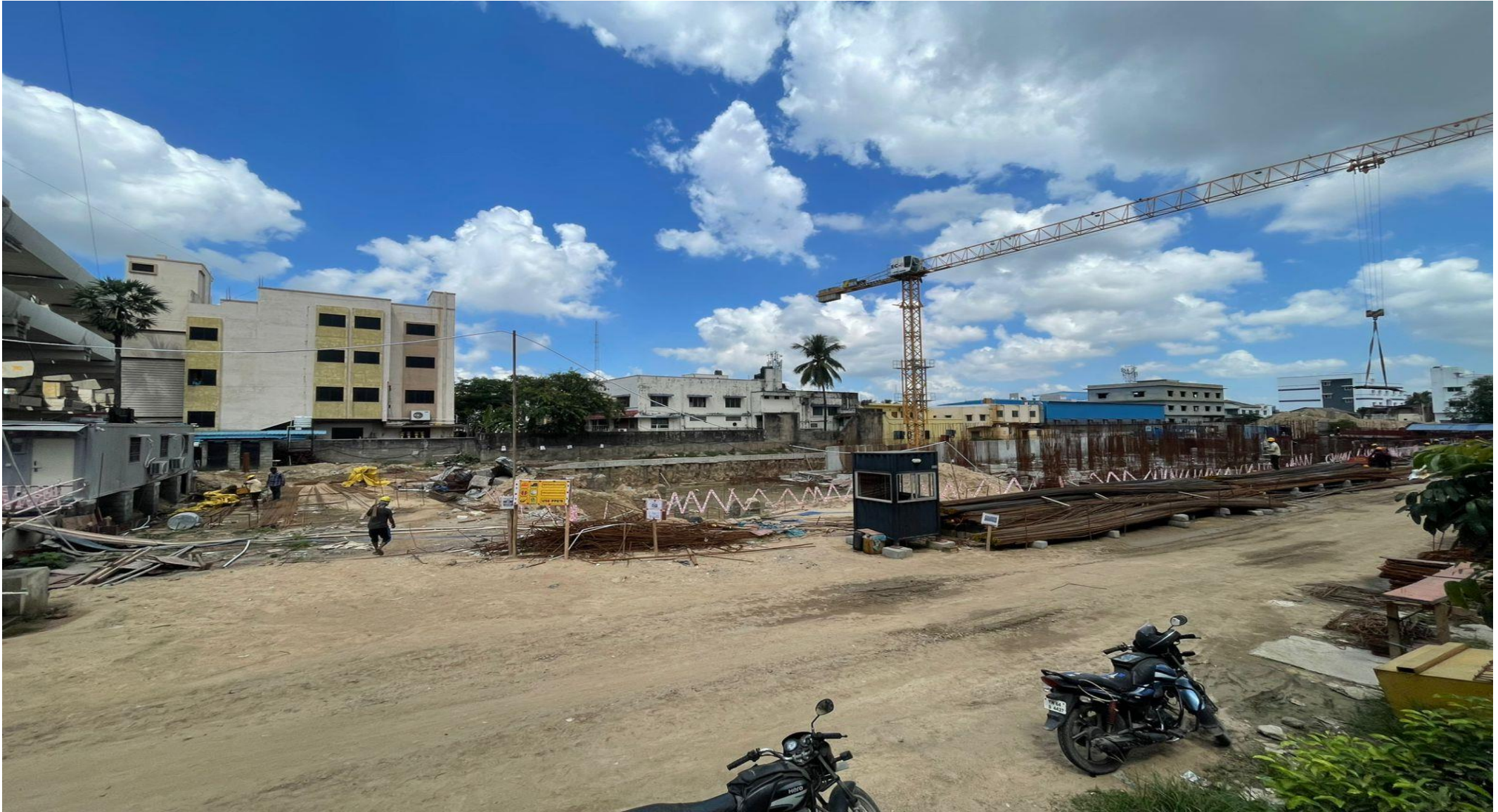
South East corner view.
