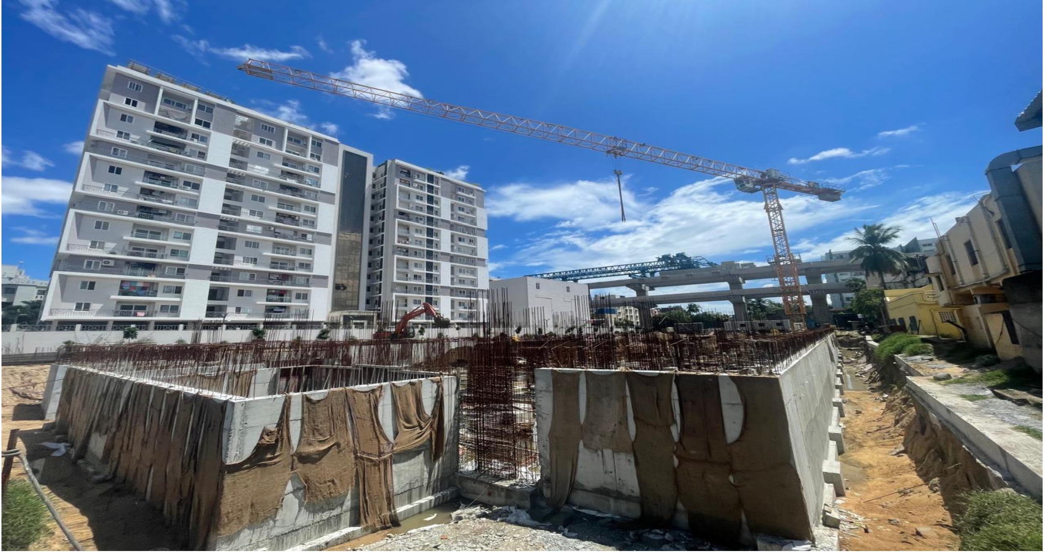
North West corner view.
