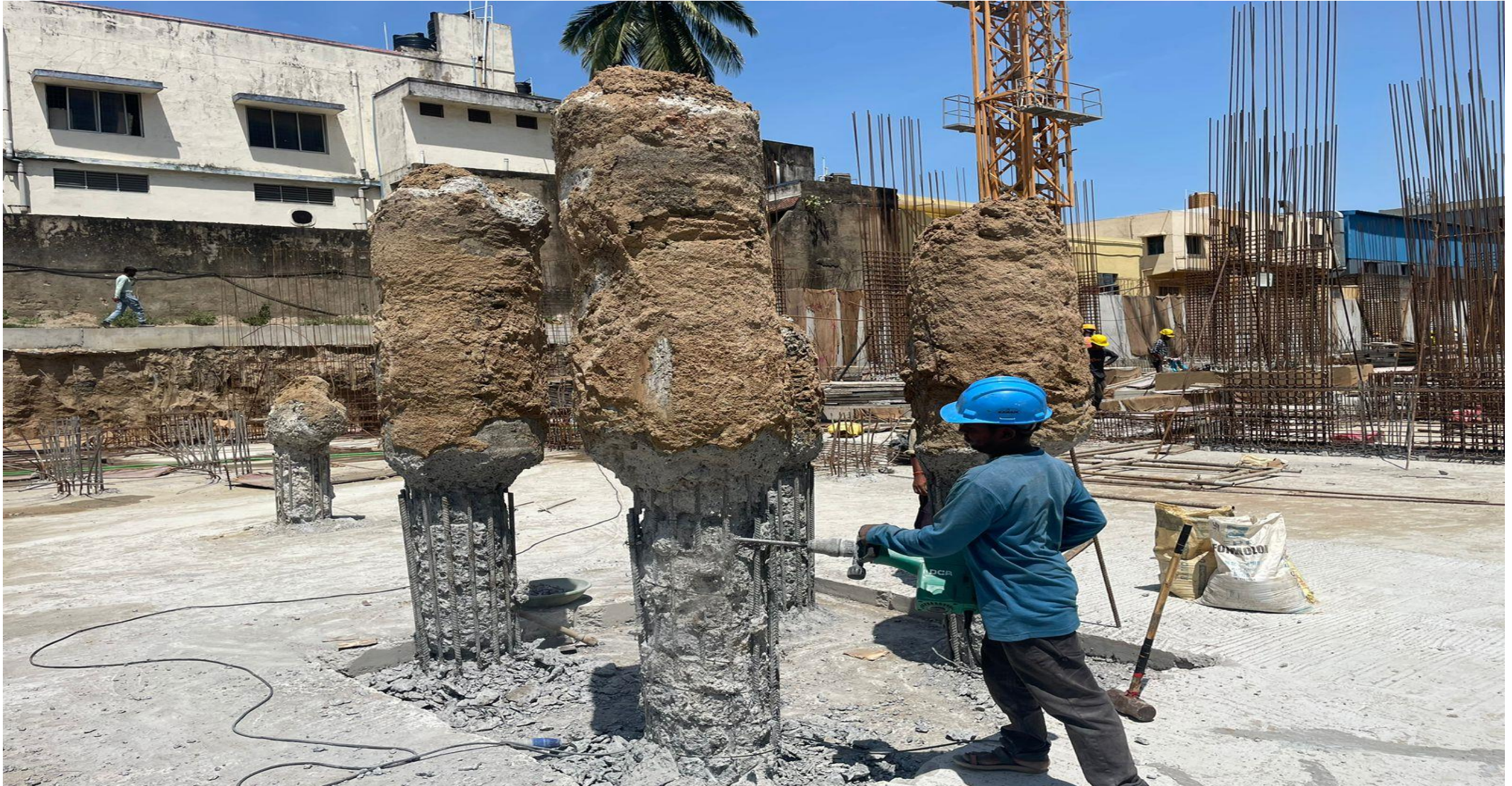
Pour-02 Pile chipping work completed.
