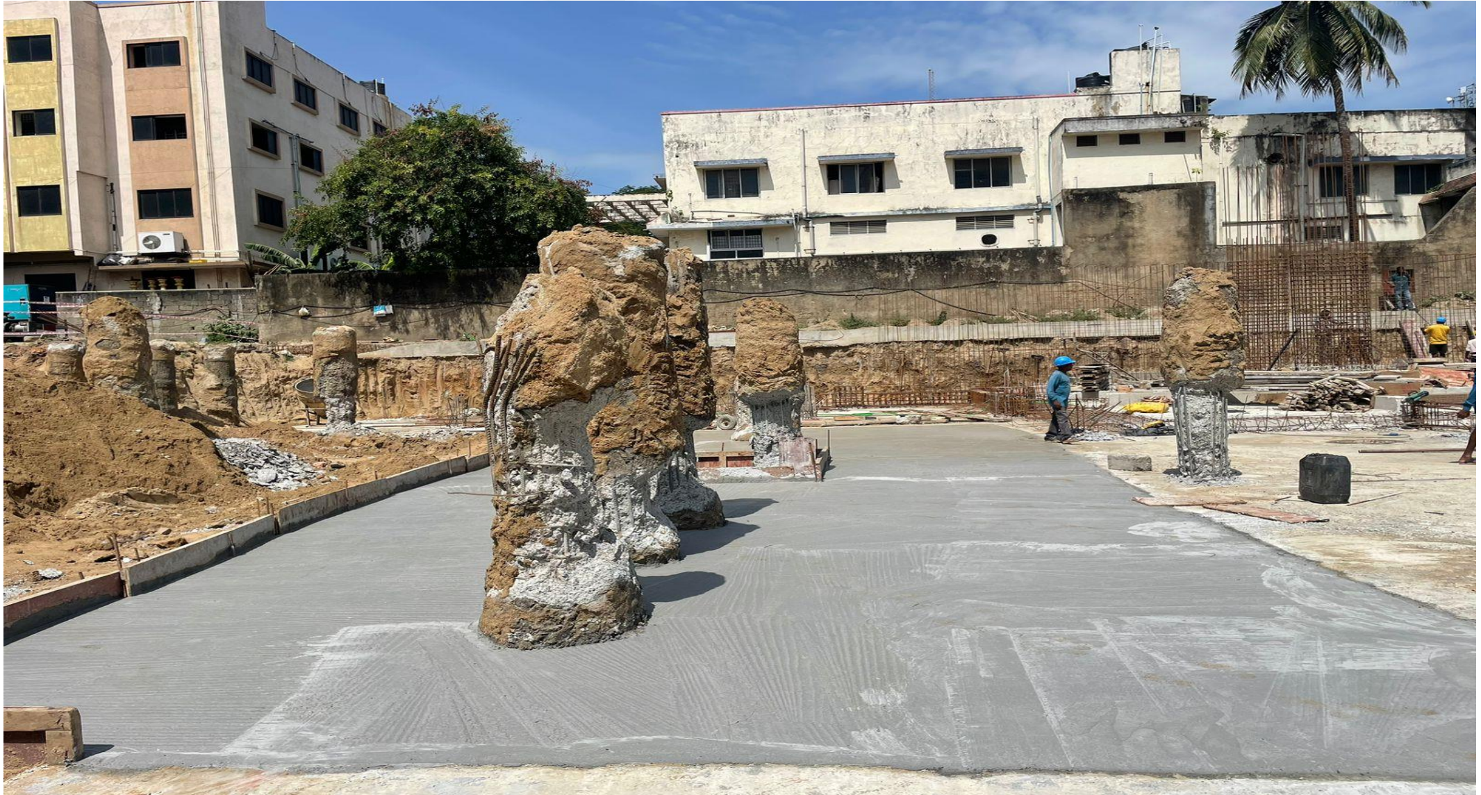
Pour-02 Remaining Area PCC work completed.
