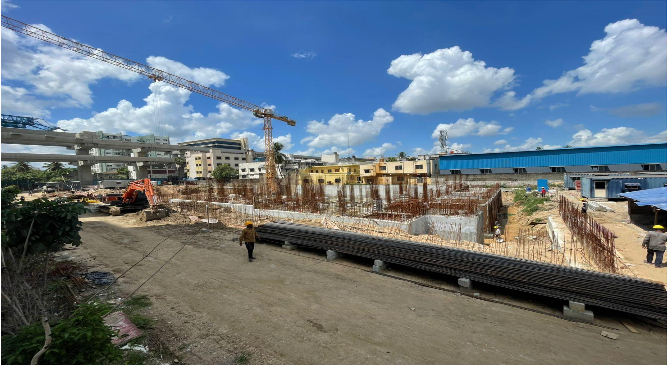
North east corner view.
