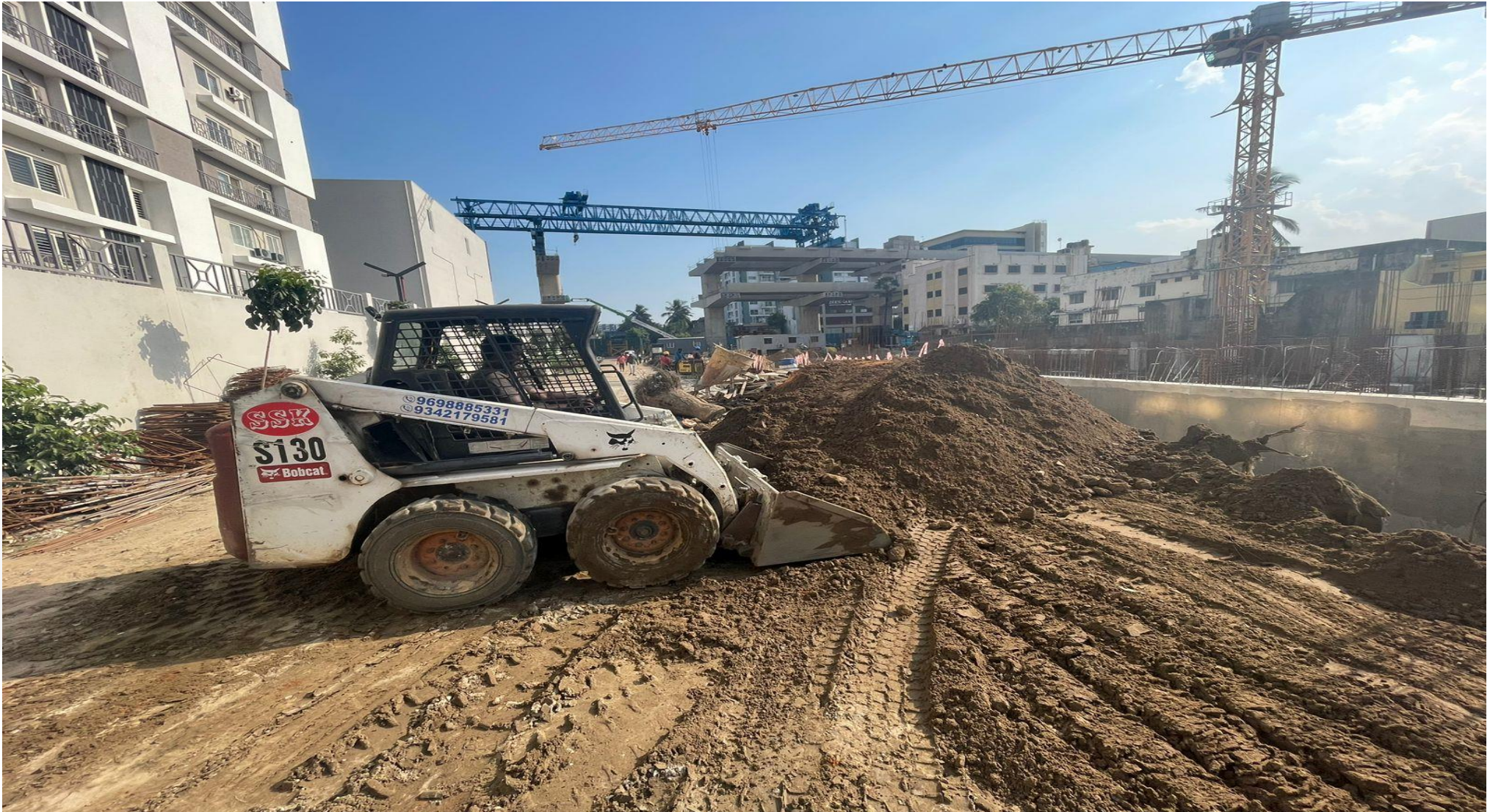
STP around area backfilling work completed.
