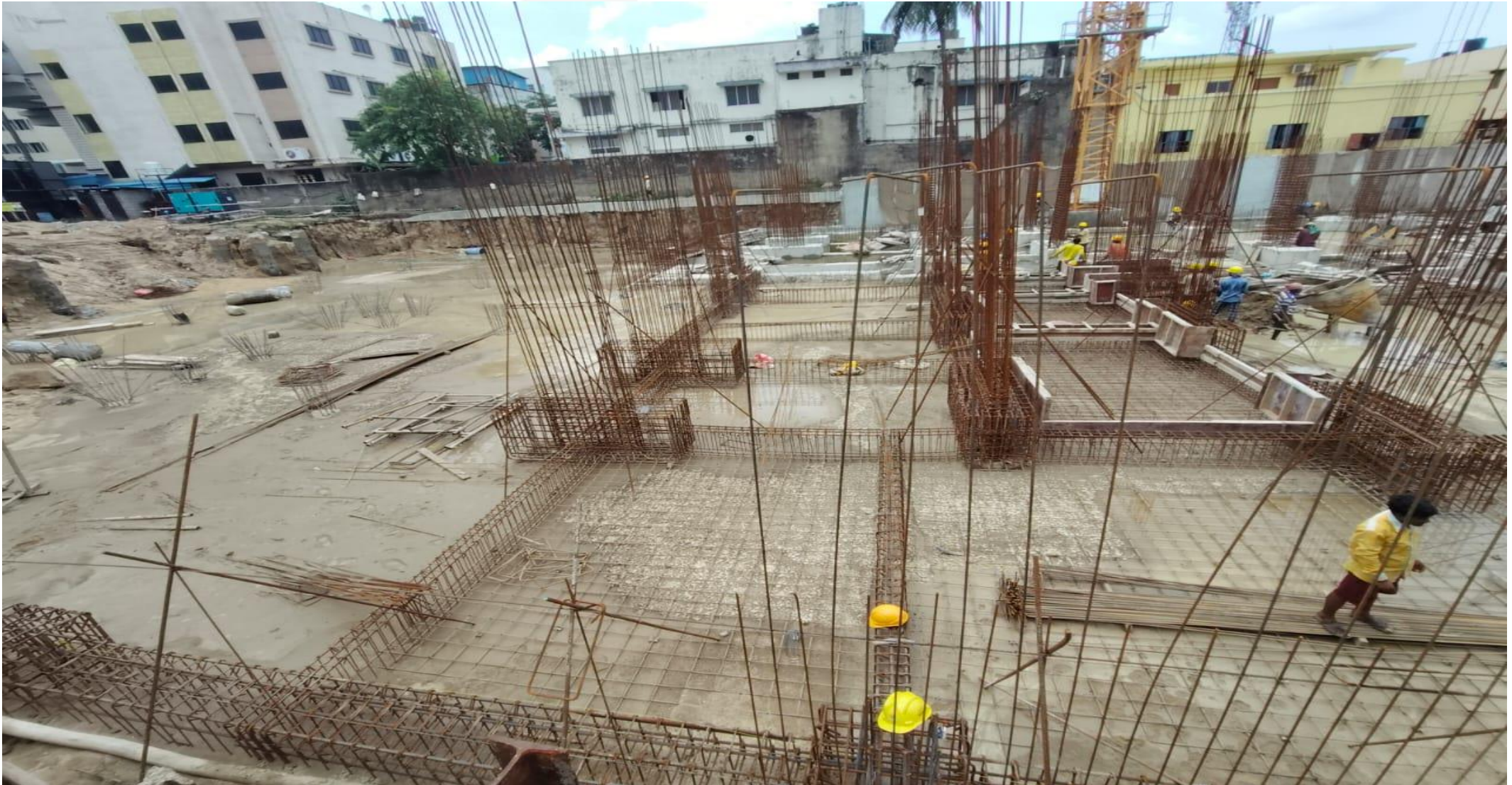
Dewatering work completed.
