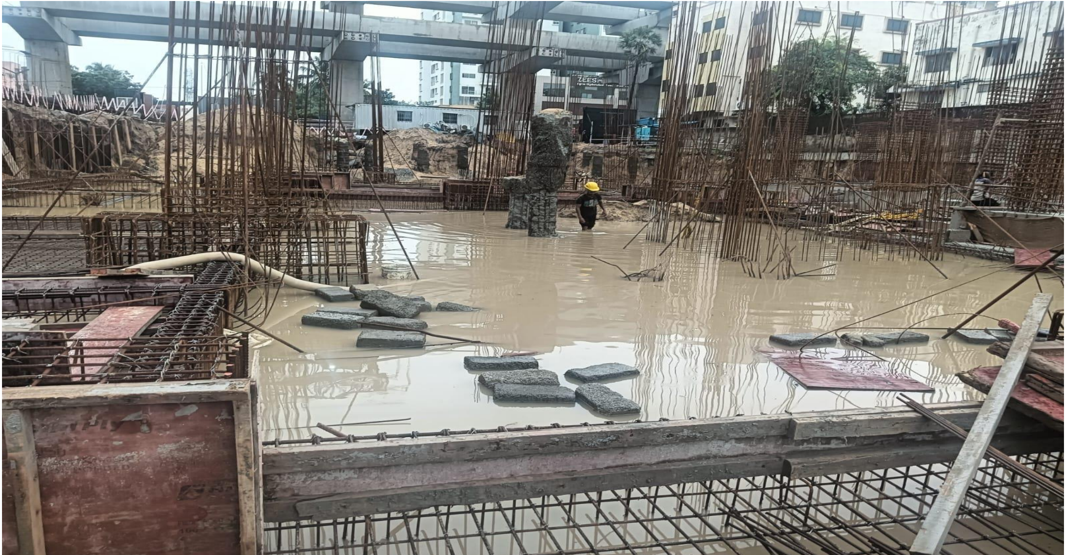
Dewatering work in progress.
