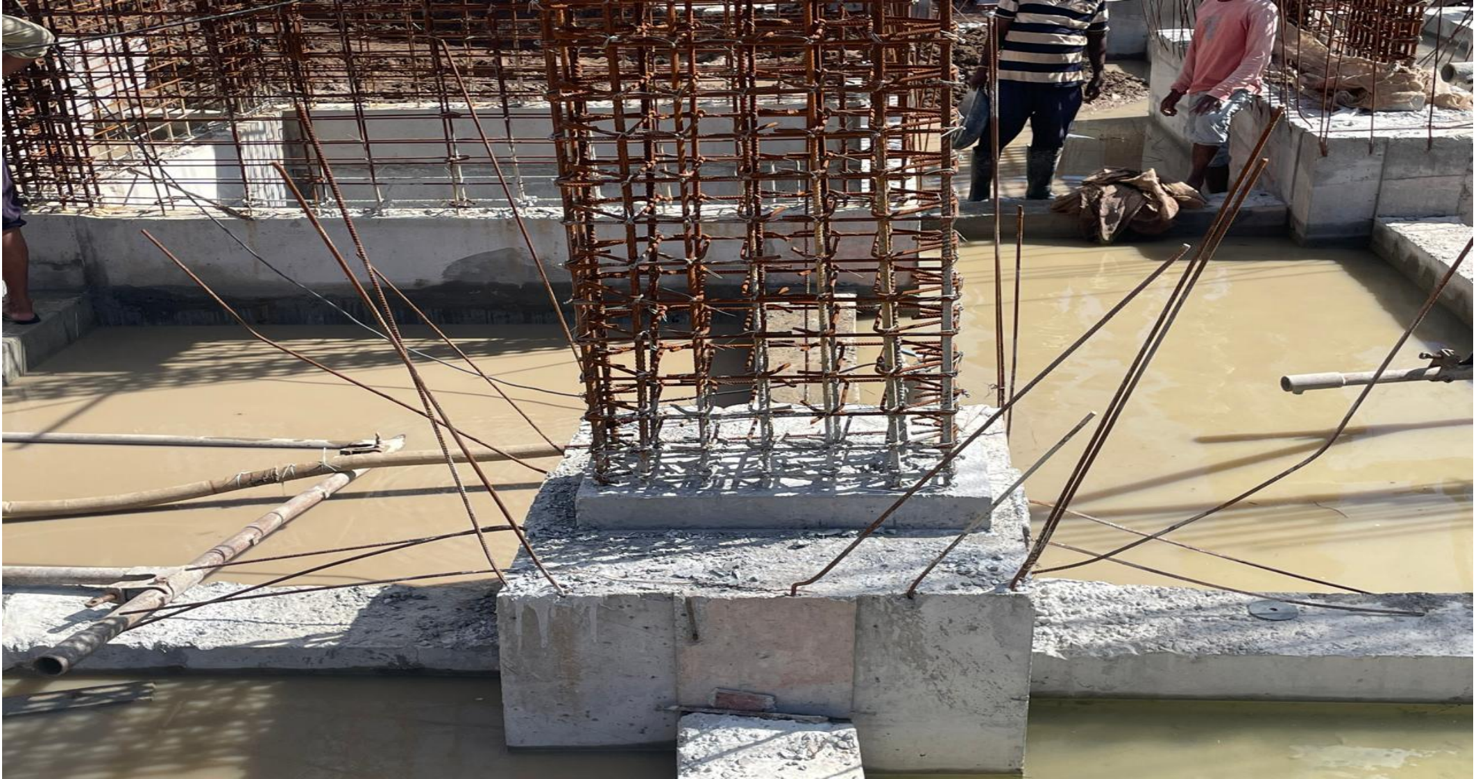
T-1 Column starter concrete work completed.
