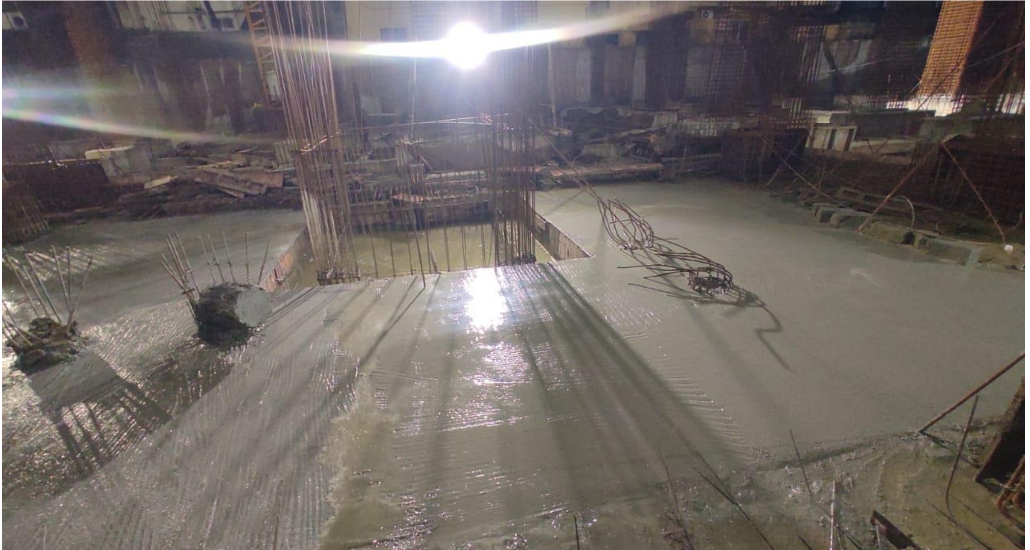
Basement floor pour-2 lift around area PCC work completed.
