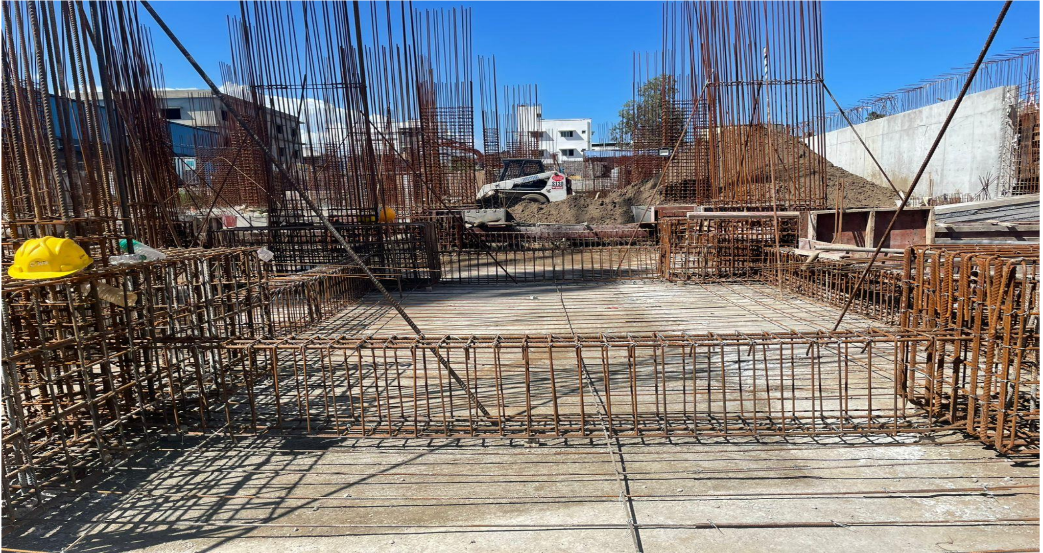
Pour 2 balance area raft slab reinforcement work in progress
