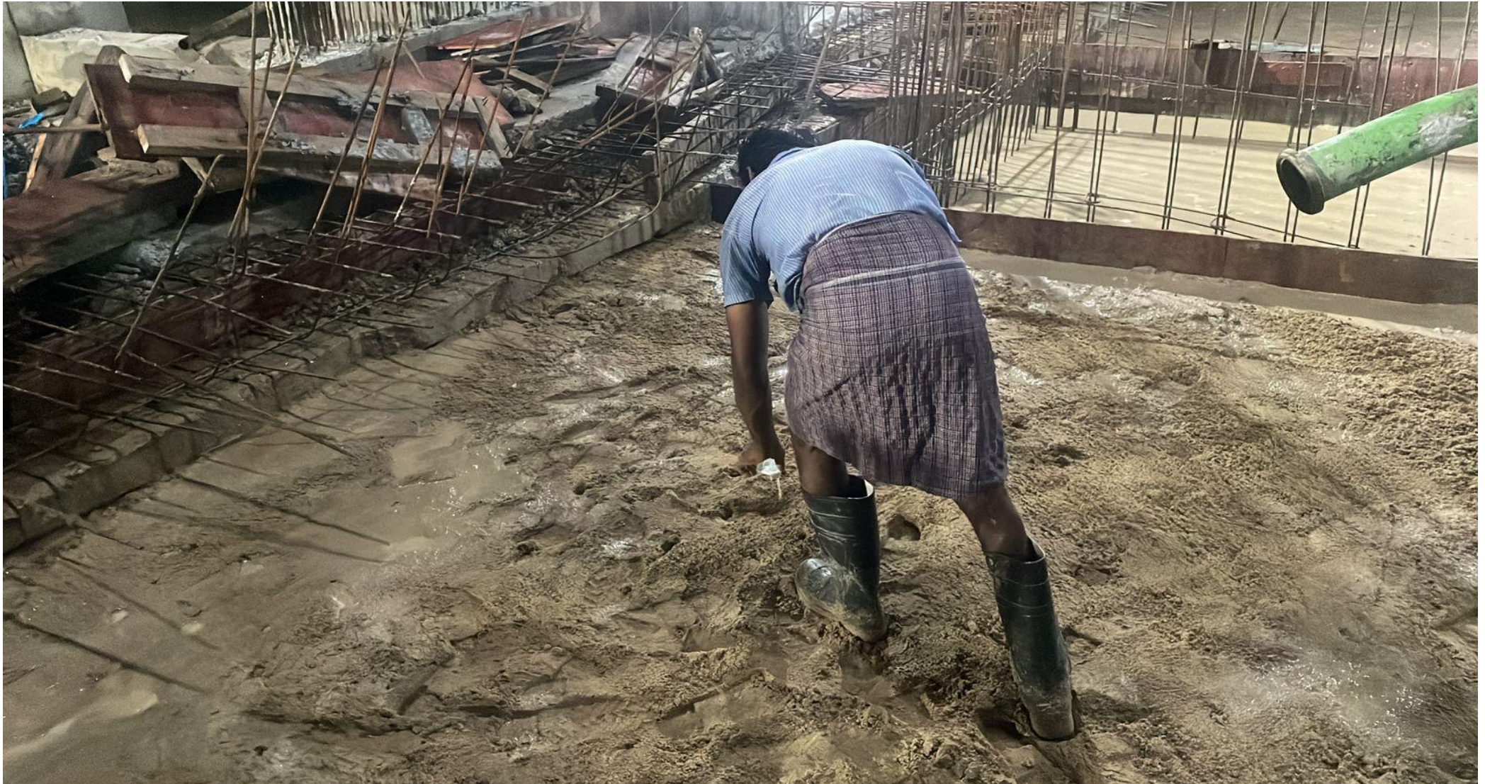
Basement floor pour-2 lift around area ATT work completed.
