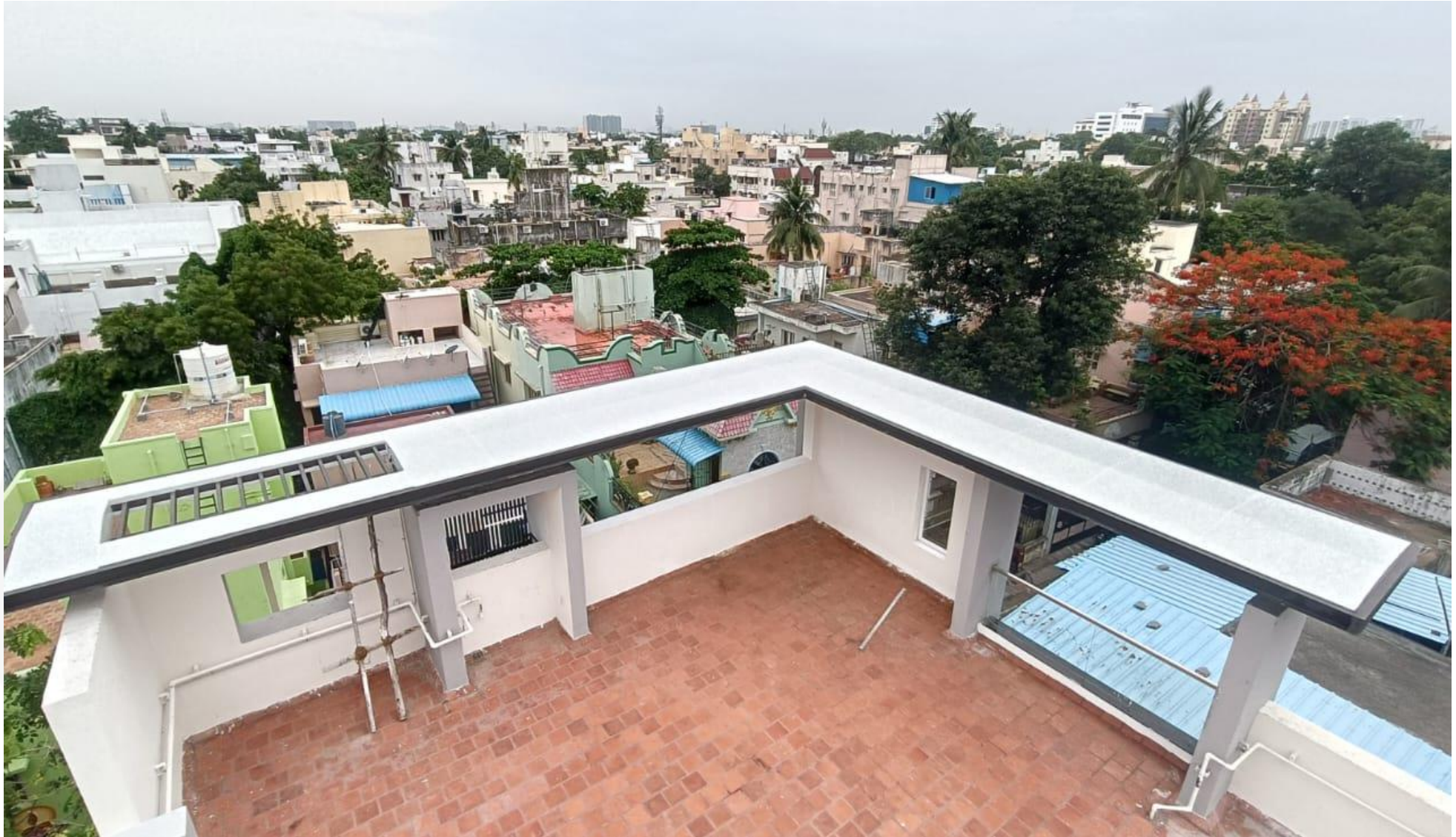
Terrace Floor Pergola ACP Cladding Work Completed
