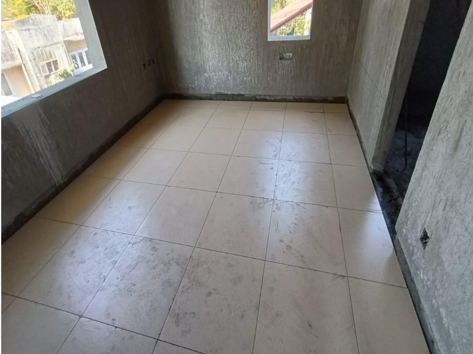
Third Floor Flooring Work In Progress
