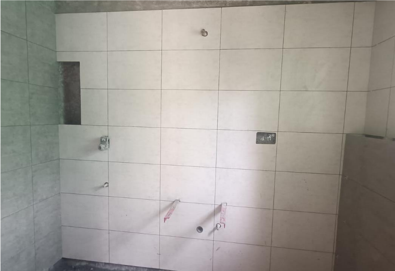
Second Floor Toilet Tiles Laying Work In Progress
