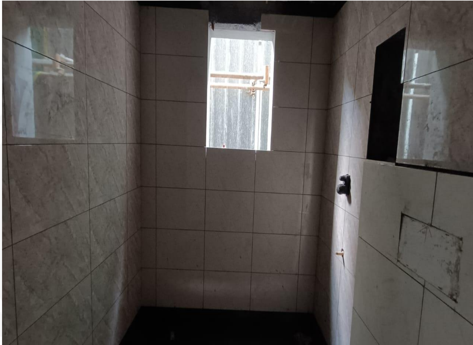
First Floor Toilet Tiles Laying Work In Progress
