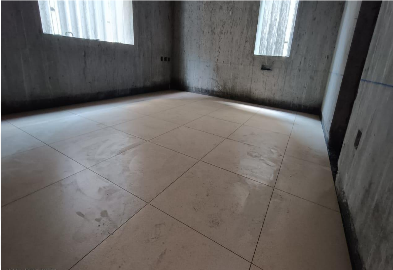
Second Floor Flooring Work In Progress
