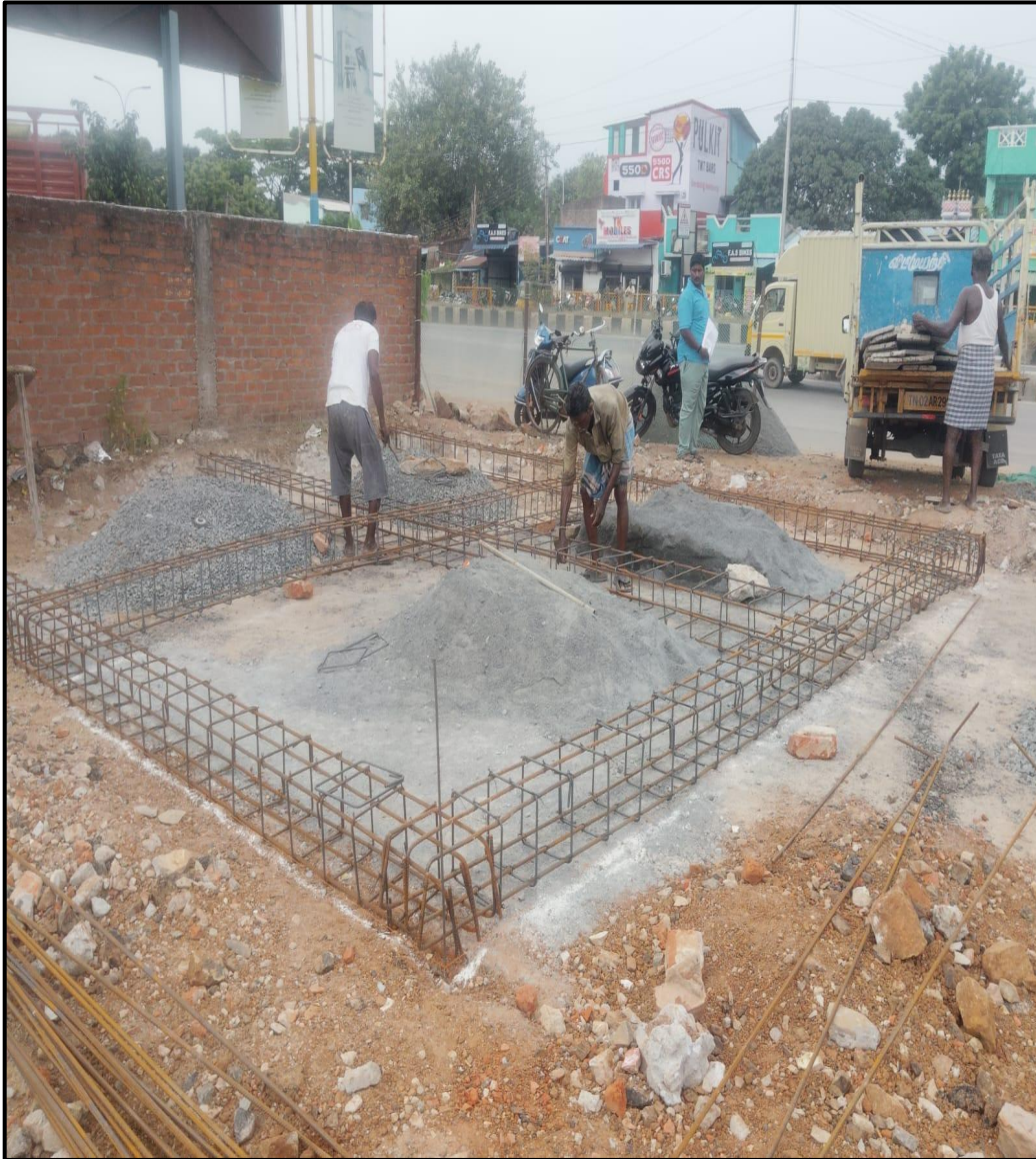
Sales Office Plinth beam Reinforcement & Shuttering work completed.
