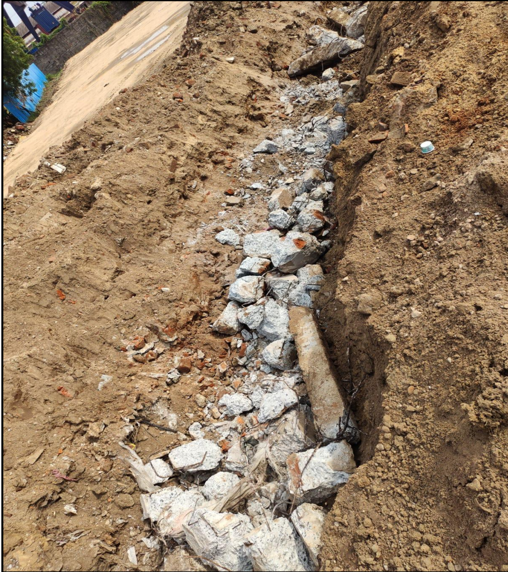
Existing Foundation demolition work in progress
