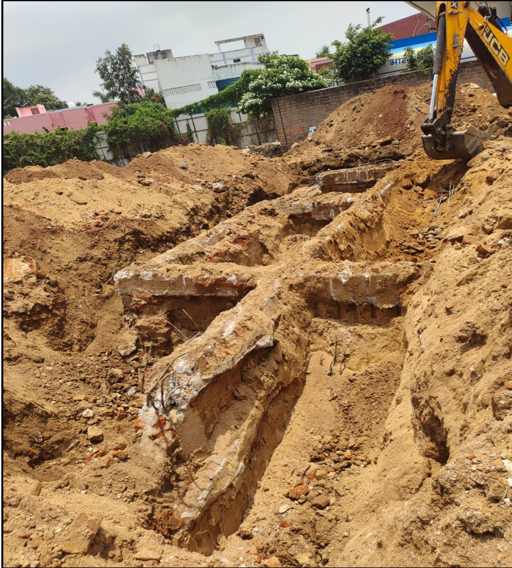
Existing Foundation demolition work in progress
