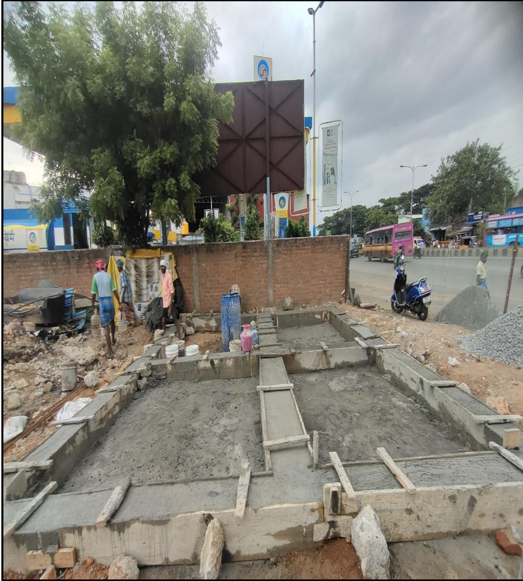
Sales Office Concrete & De-shuttering work completed.
