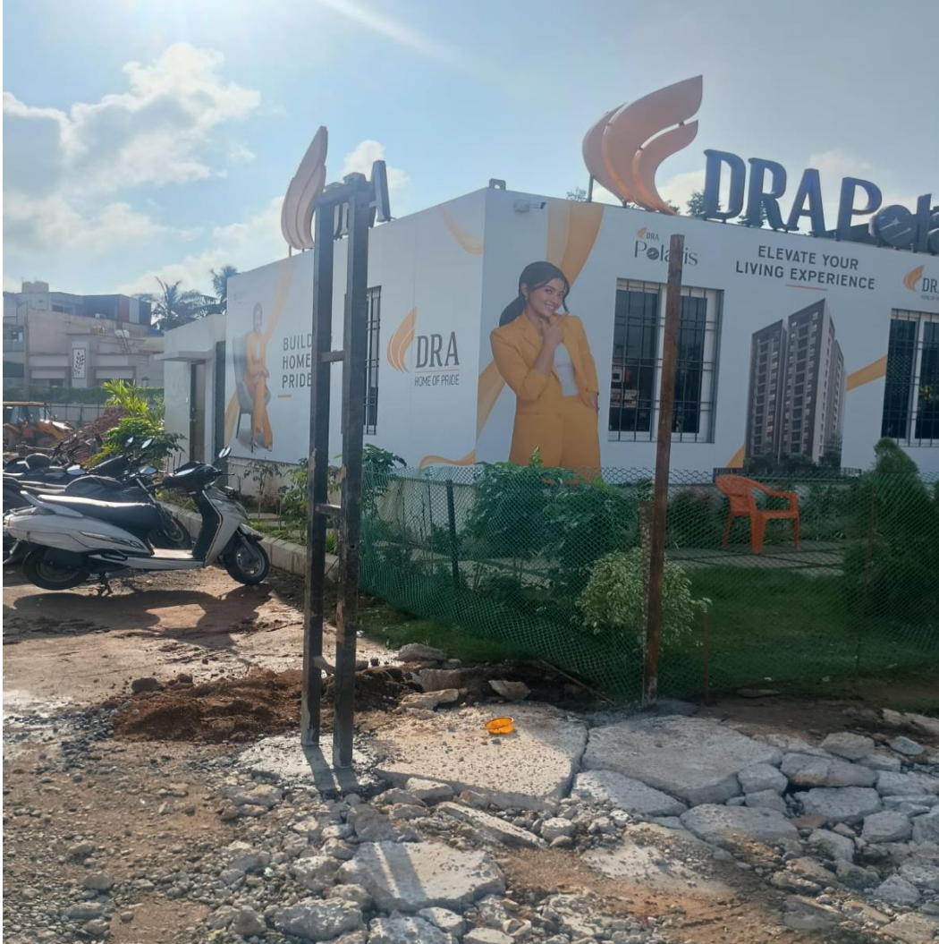
Temporary Gate vertical post concrete work completed
