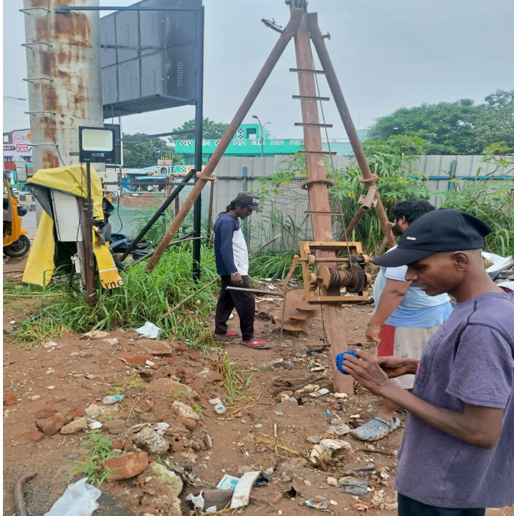
Compound wall pile boring commencement work in progress
