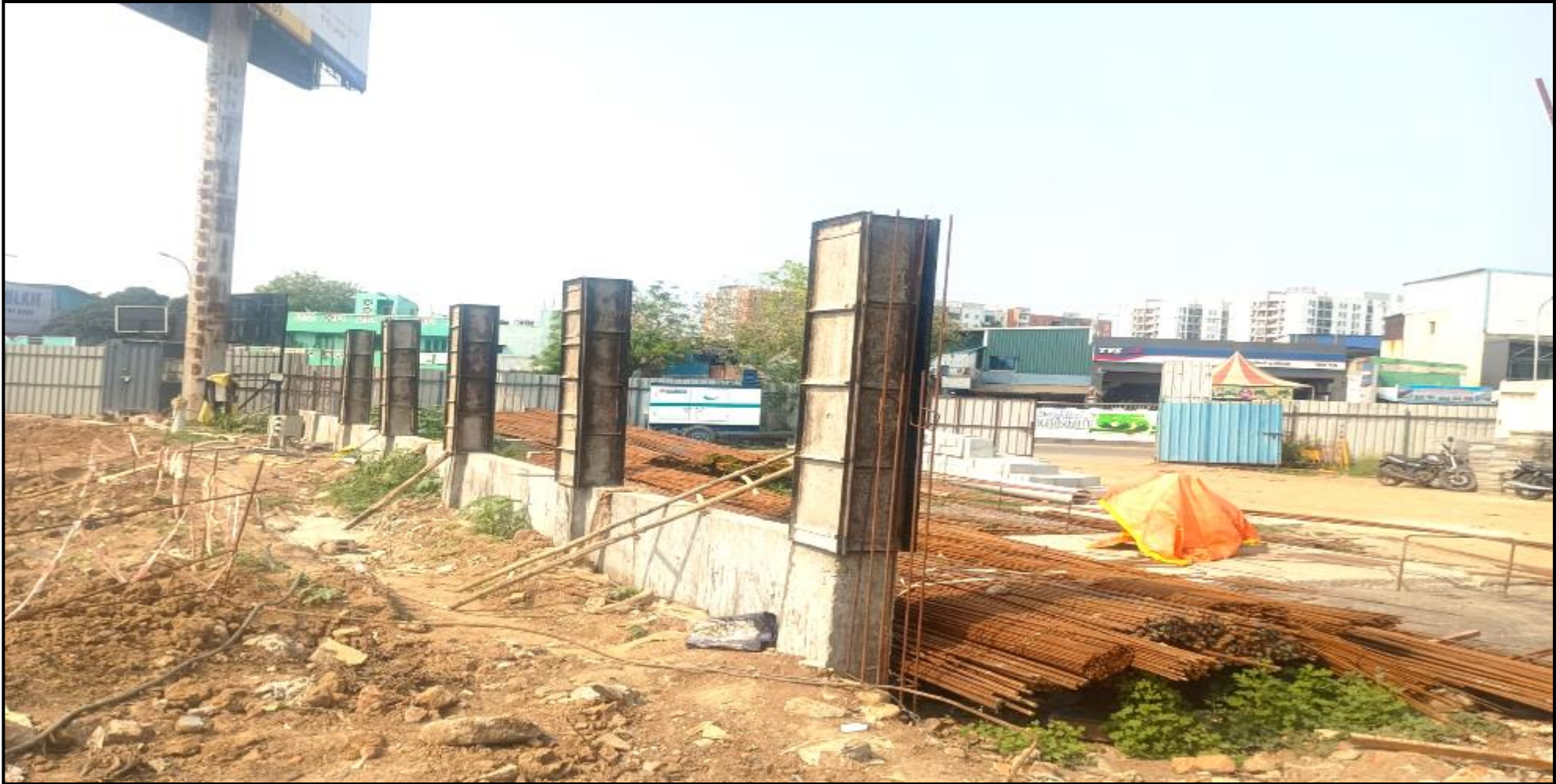
Compound wall – Column concrete above RC wall (5/52 no's) completed
