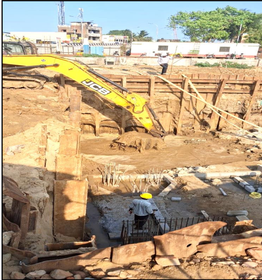
UG Sump – Excavation work completed (1500/1500 cum)
