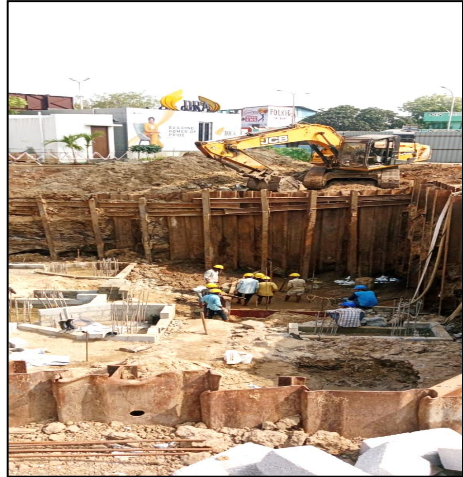
UG Sump – Excavation work completed (1500/1500 cum)
