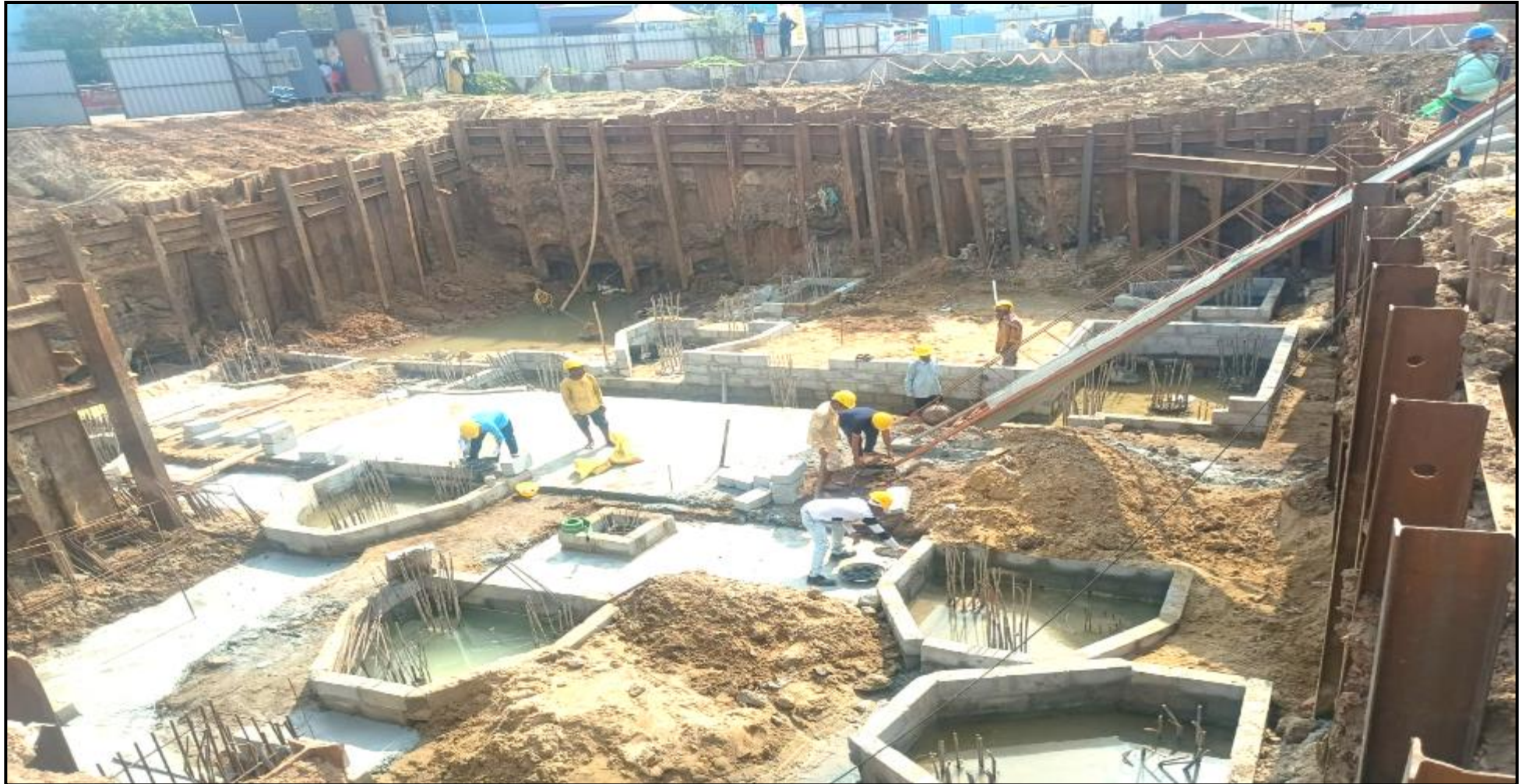
UG Sump & Main building – Pile cap block work (49/65 no's) completed
