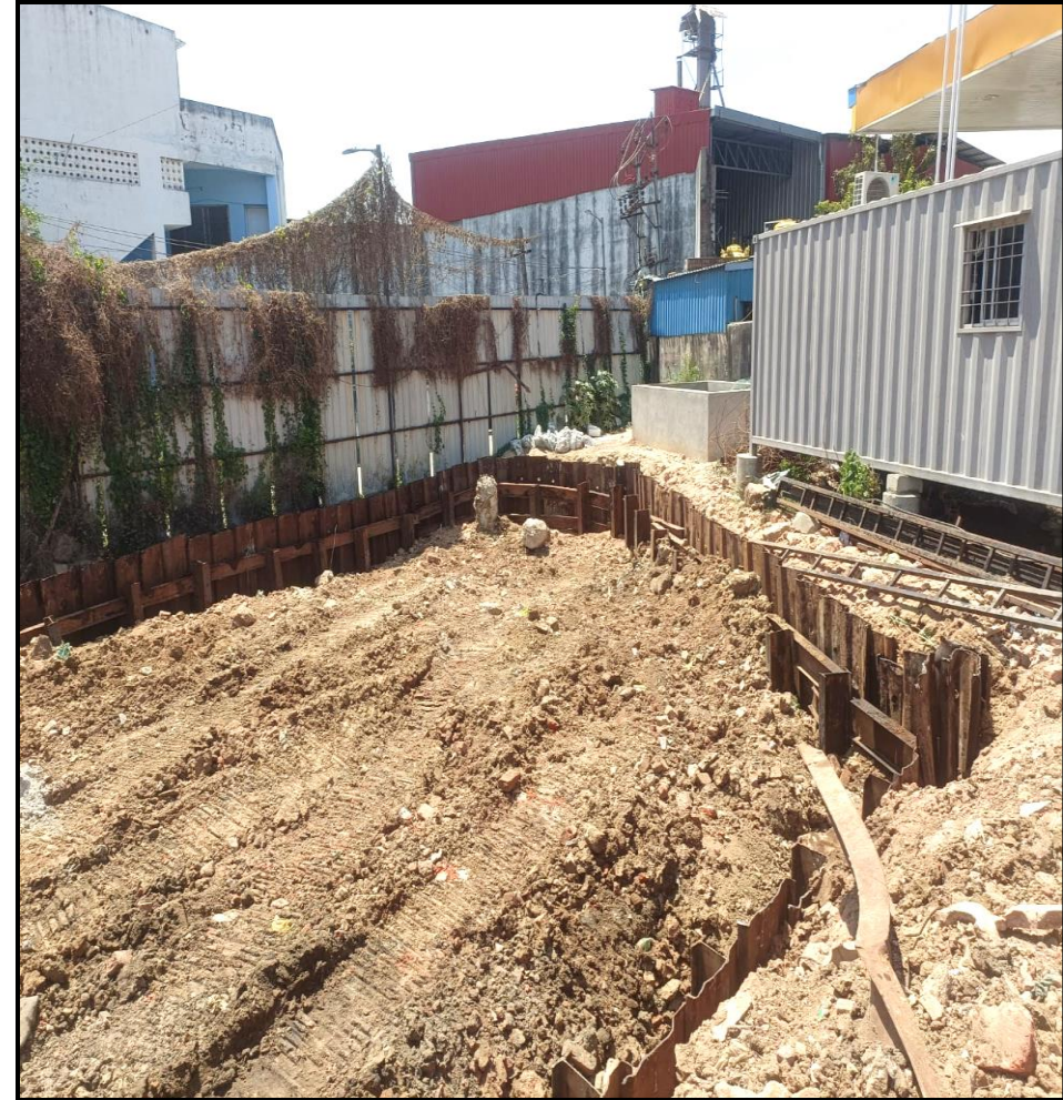
STP – Shoring work completed (74.5/74.5m)
