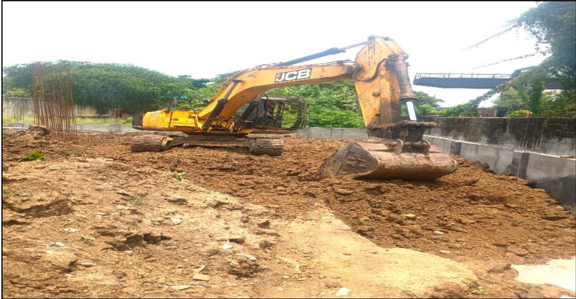
Compound wall – Soil back filling work at south side wall
