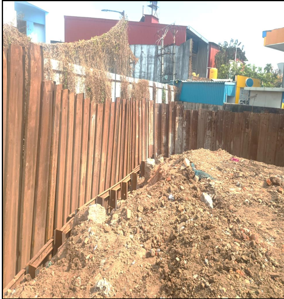
STP – Shoring work completed (74.5/74.5m)
