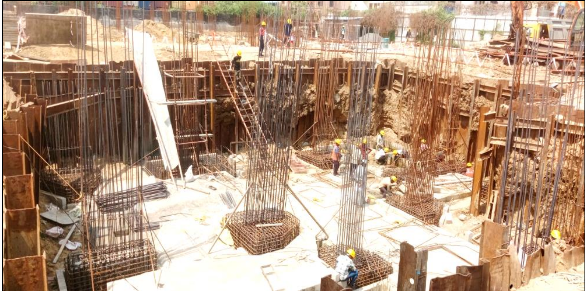
UG Sump – Pile cap reinforcement work (12/18 no's) completed
