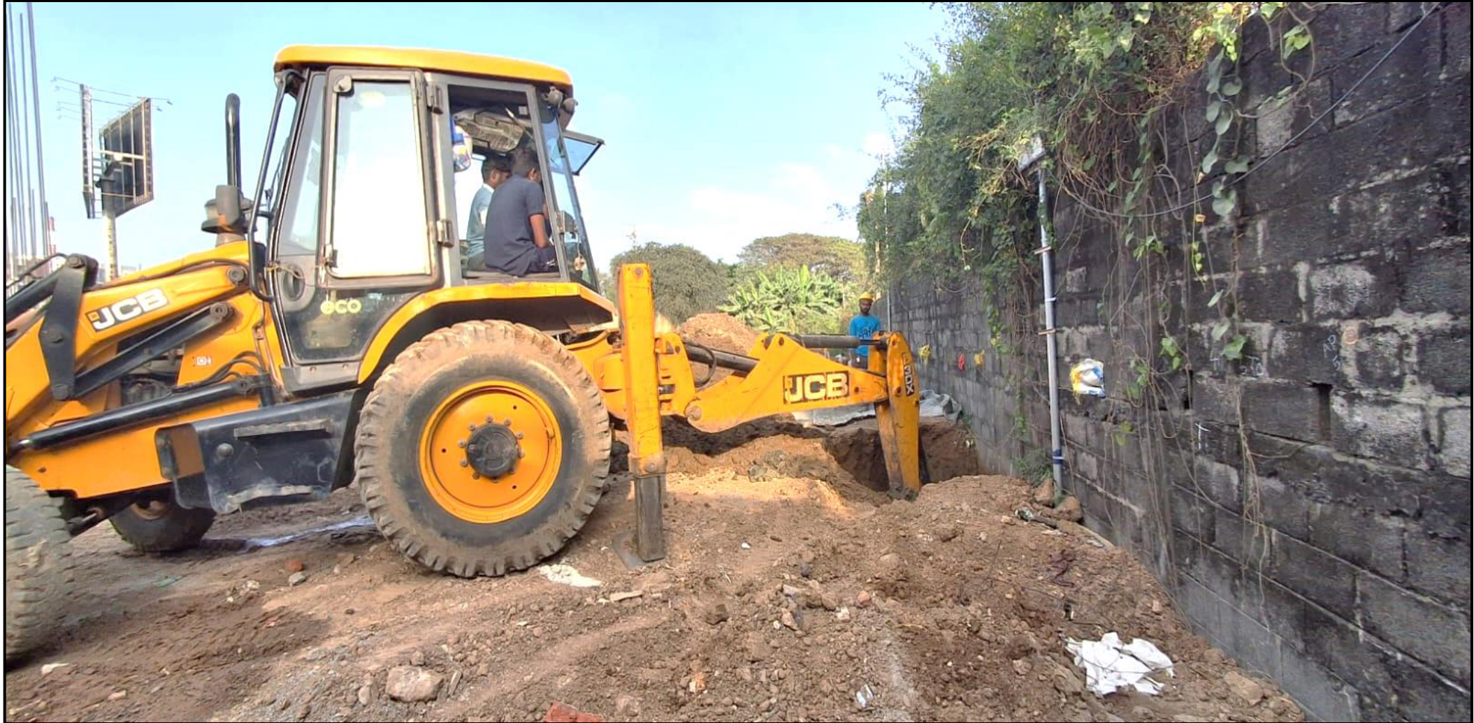
Compound wall – Excavation work in progress (26/29 nos completed)
