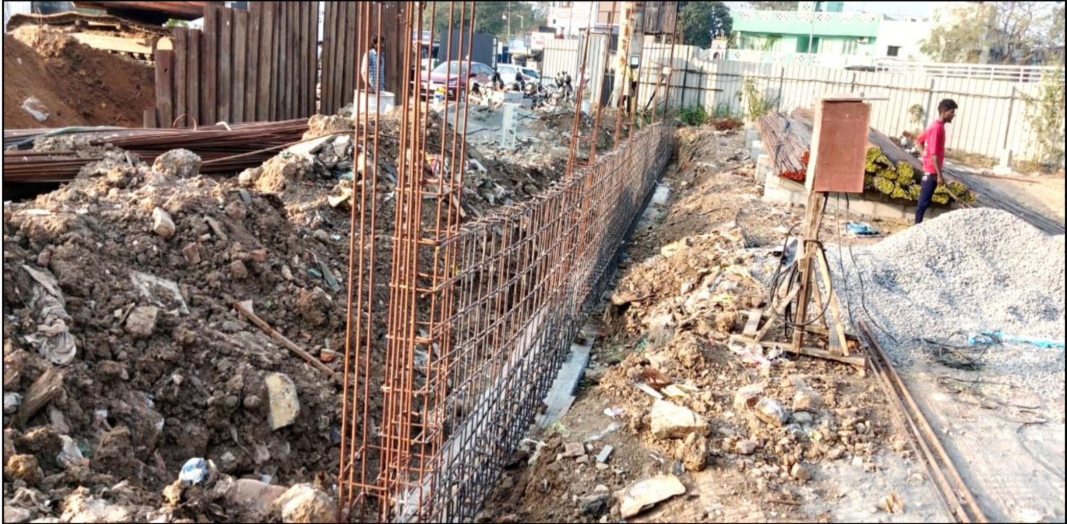
Compound wall – Plinth beam & RC wall reinforcement work 41/113m completed
