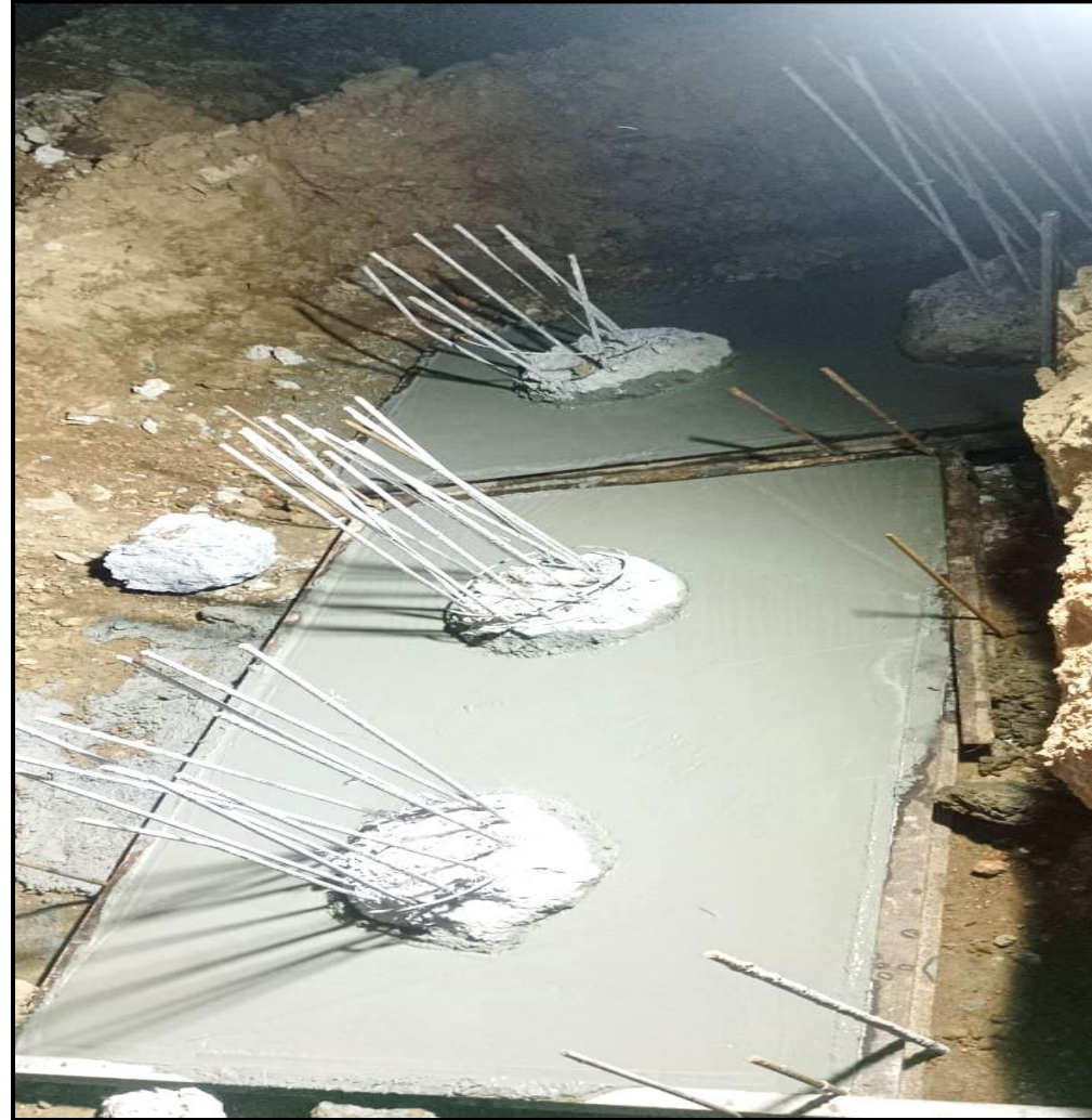
Main building – Pile cap PCC laying work in progress ( 32/47 no's completed)
