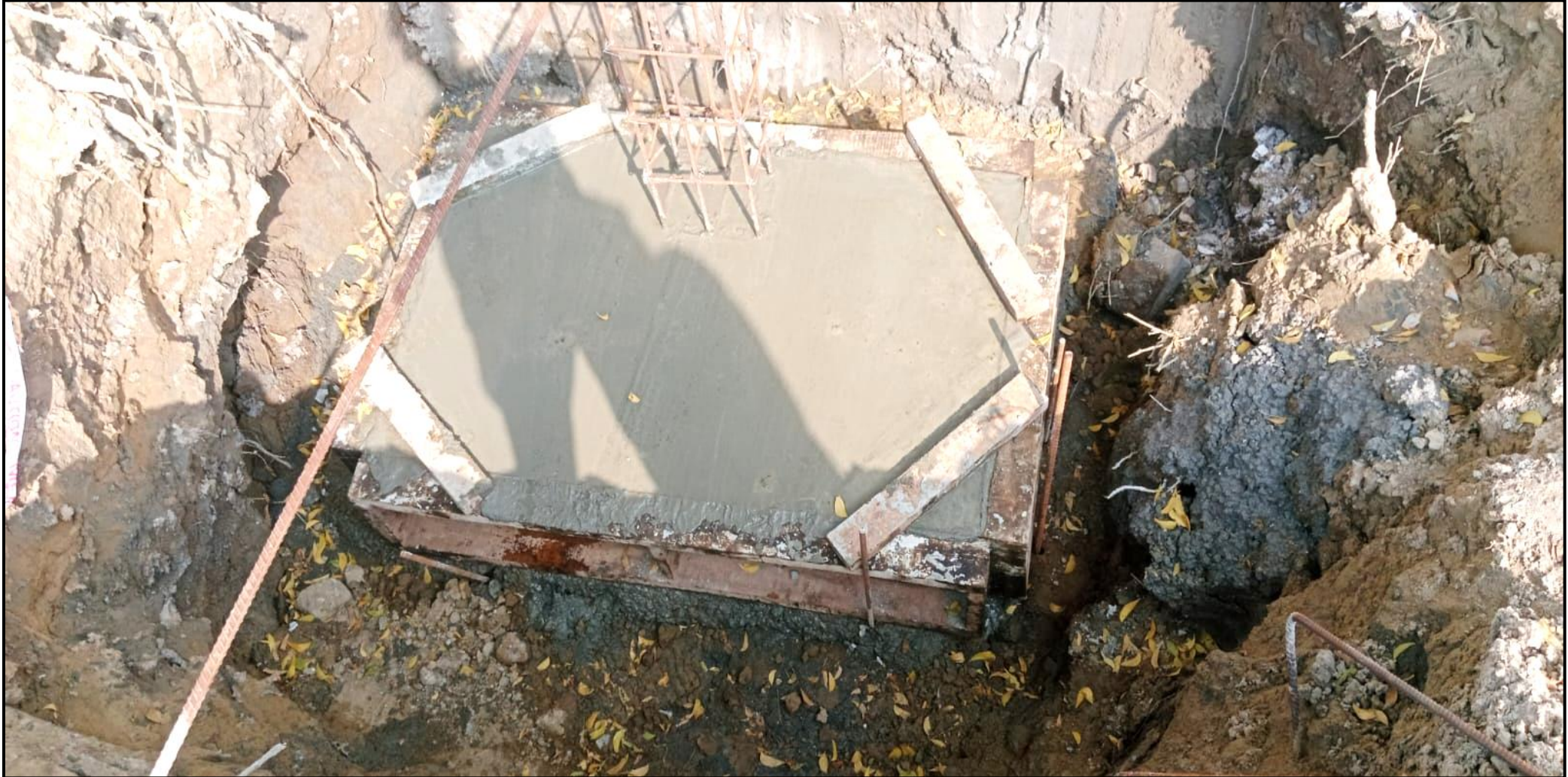
Compound wall - Footing concrete 19/29 no's completed
