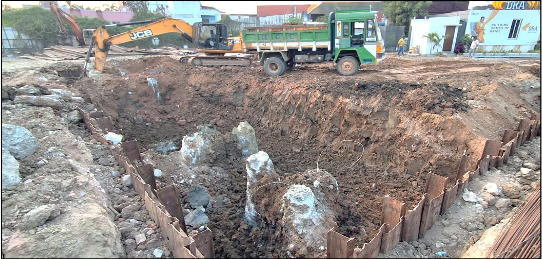
UG Sump – Excavation work in progress (500cum excavated)
