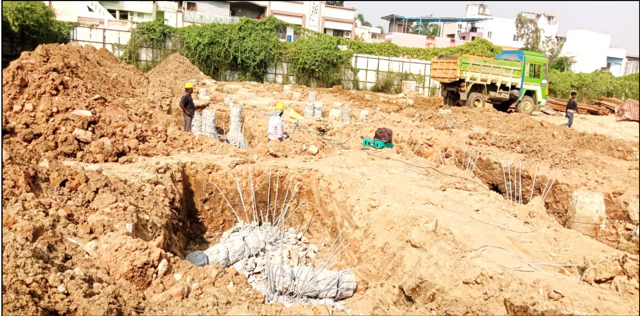
Main Building – Pile cap chipping work in progress (85/126 Nos completed)
