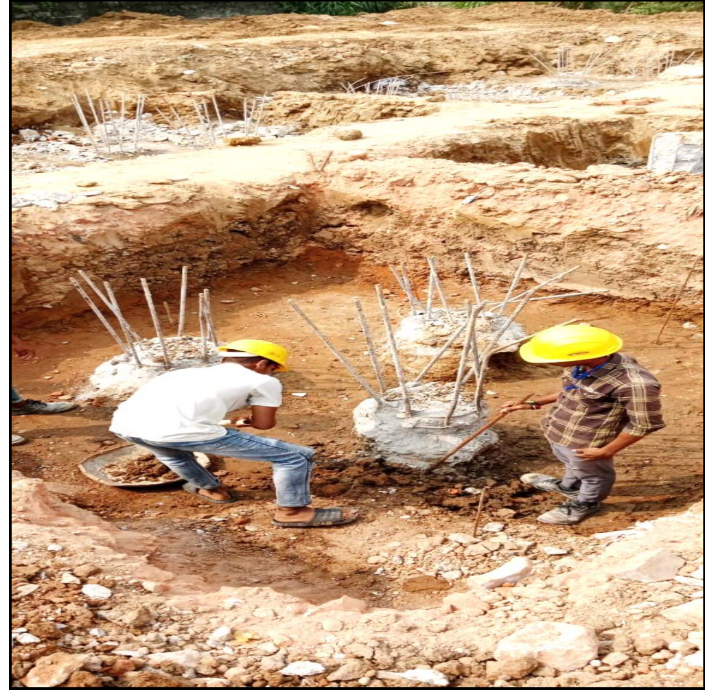
Main Building – Pile cap dressing work in progress (32/47 no's Completed)
