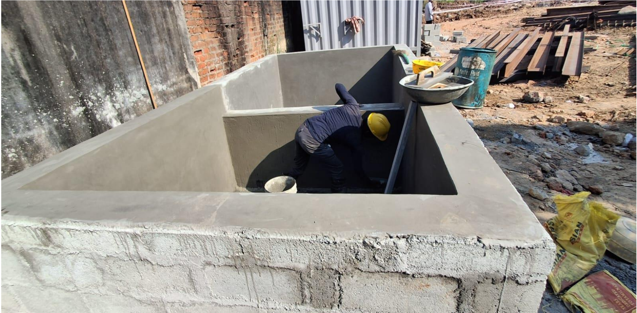
Curing tank internal & external plastering work completed
