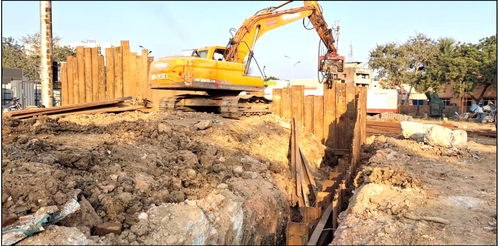
Main building – UG sump shoring work (80.5/80.5m completed)
