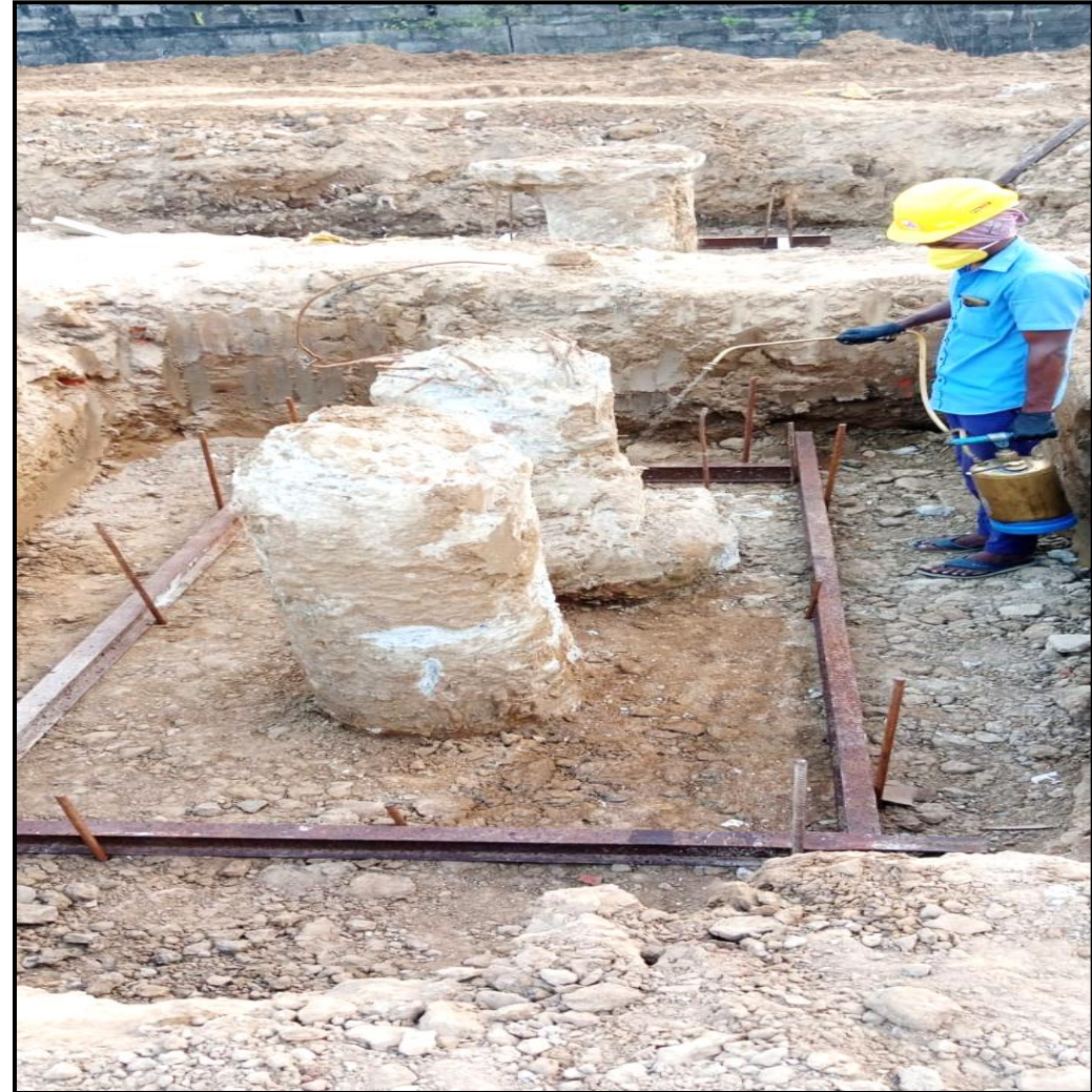
Main Building – Pile cap ATT work in progress (32/47 no's completed)
