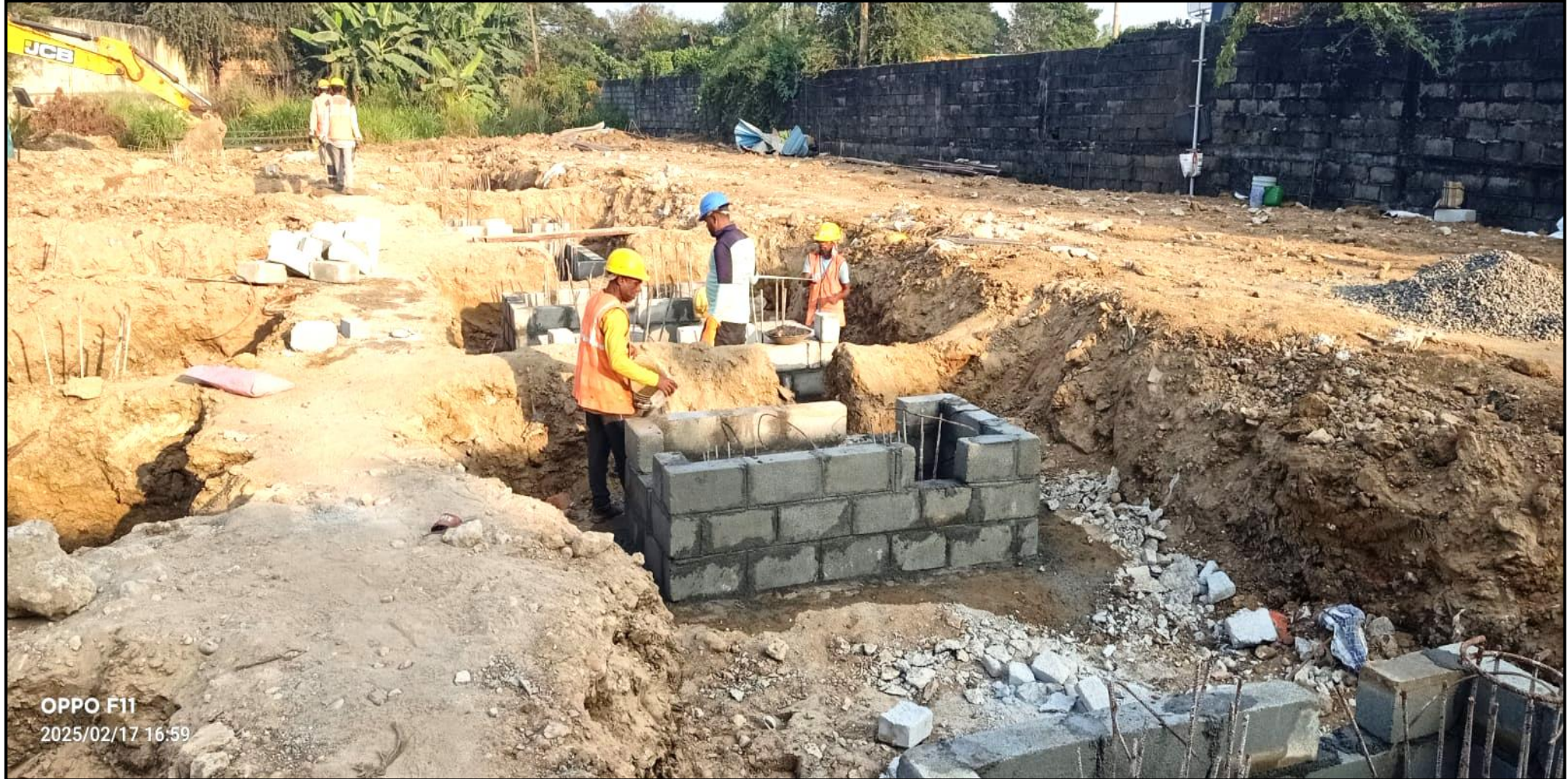
Main building – Pile cap block work in progress (29/47 no's completed)
