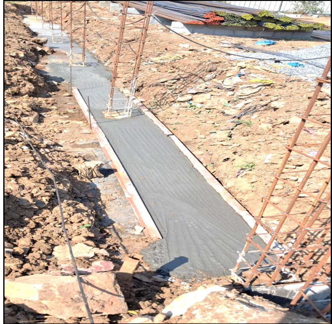
Compound wall – Plinth beam PCC 55/113m completed
