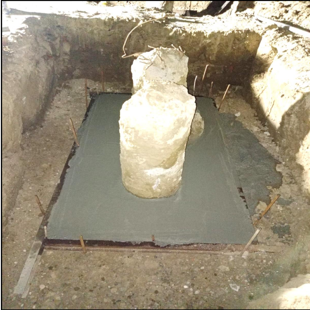
Main building – Pile cap PCC laying work in progress ( 32/47 no's completed)
