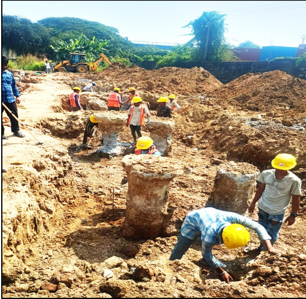
Main Building – Pile cap dressing work in progress (32/47 no's Completed)
