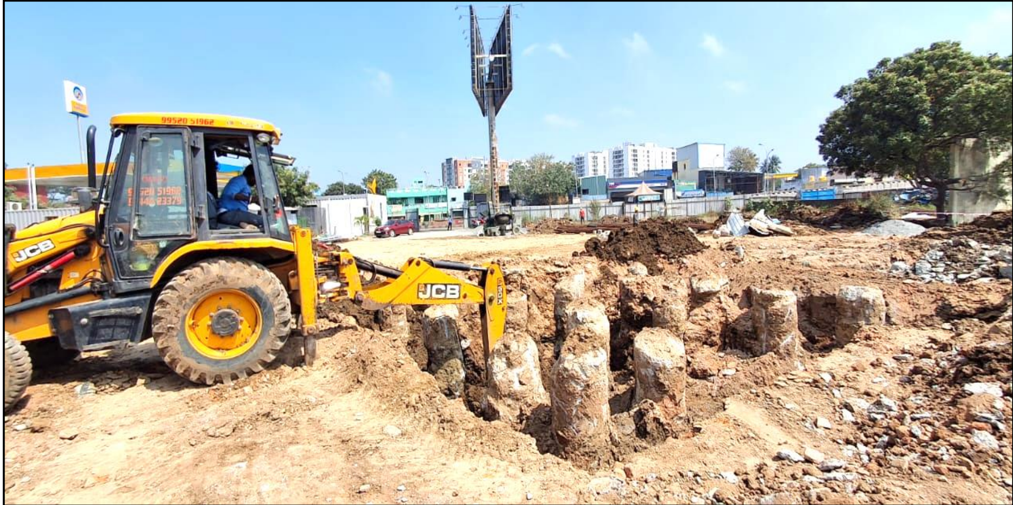
Main Building – Pile cap excavation work in progress (34/47 no's completed)
