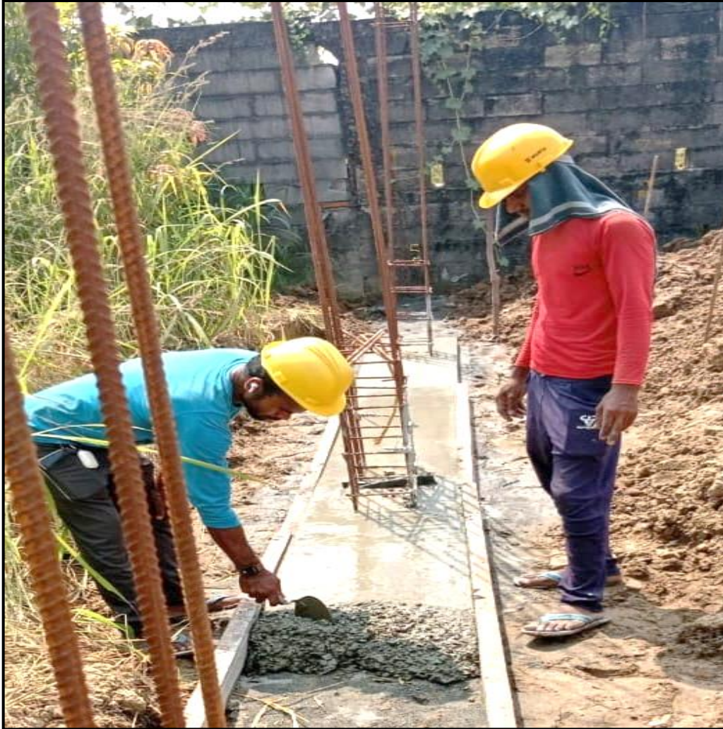
Compound wall – Plinth beam PCC 55/113m completed
