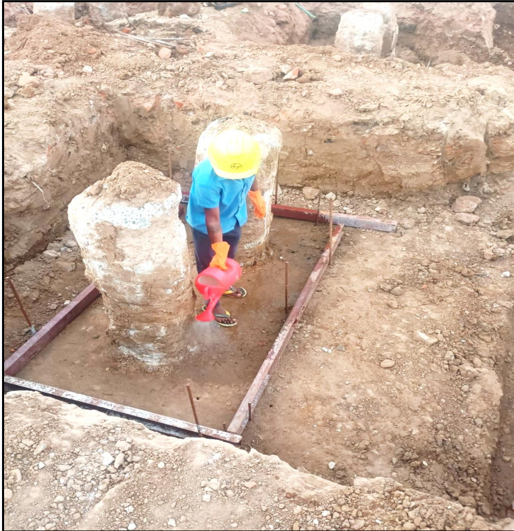
Main Building – Pile cap ATT work in progress (32/47 no's completed)
