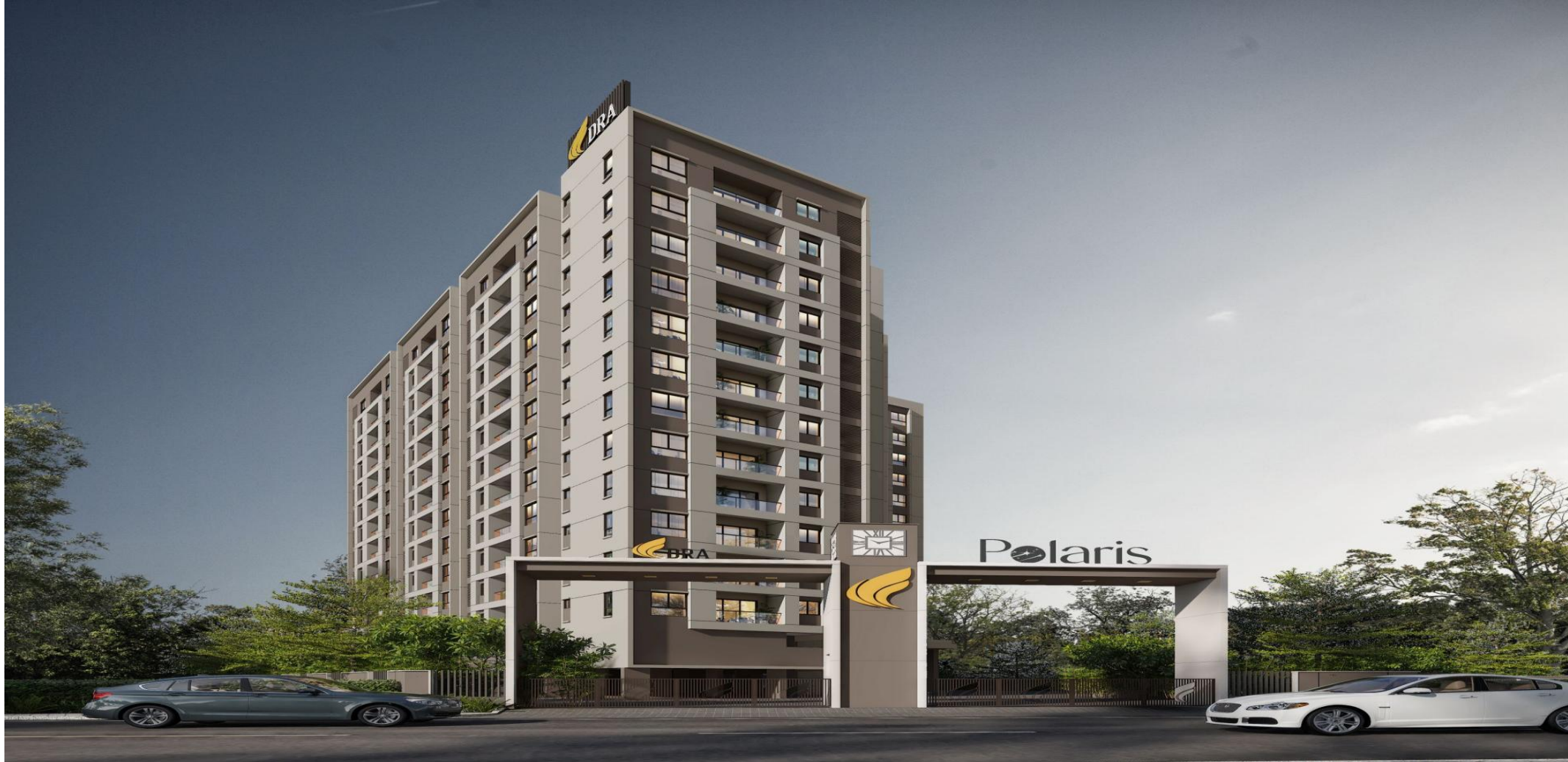
DRA POLARIS Construction updates photos – January 2025
