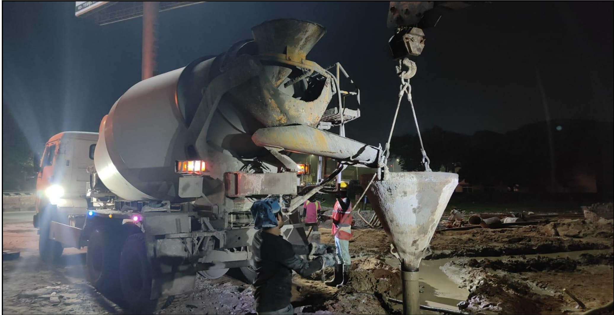
DRA Polaris - Piling concrete work completed- 220/220 Nos completed
