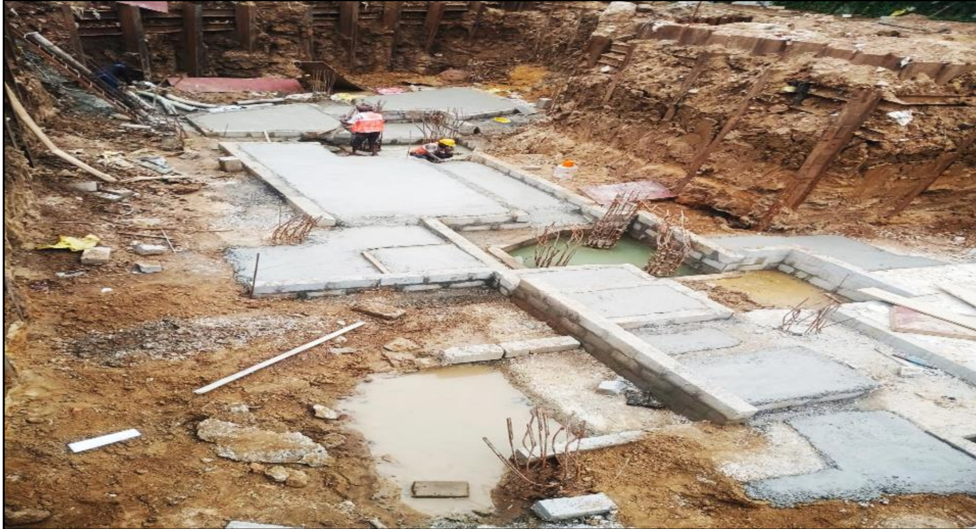
STP – Raft pcc work completed
