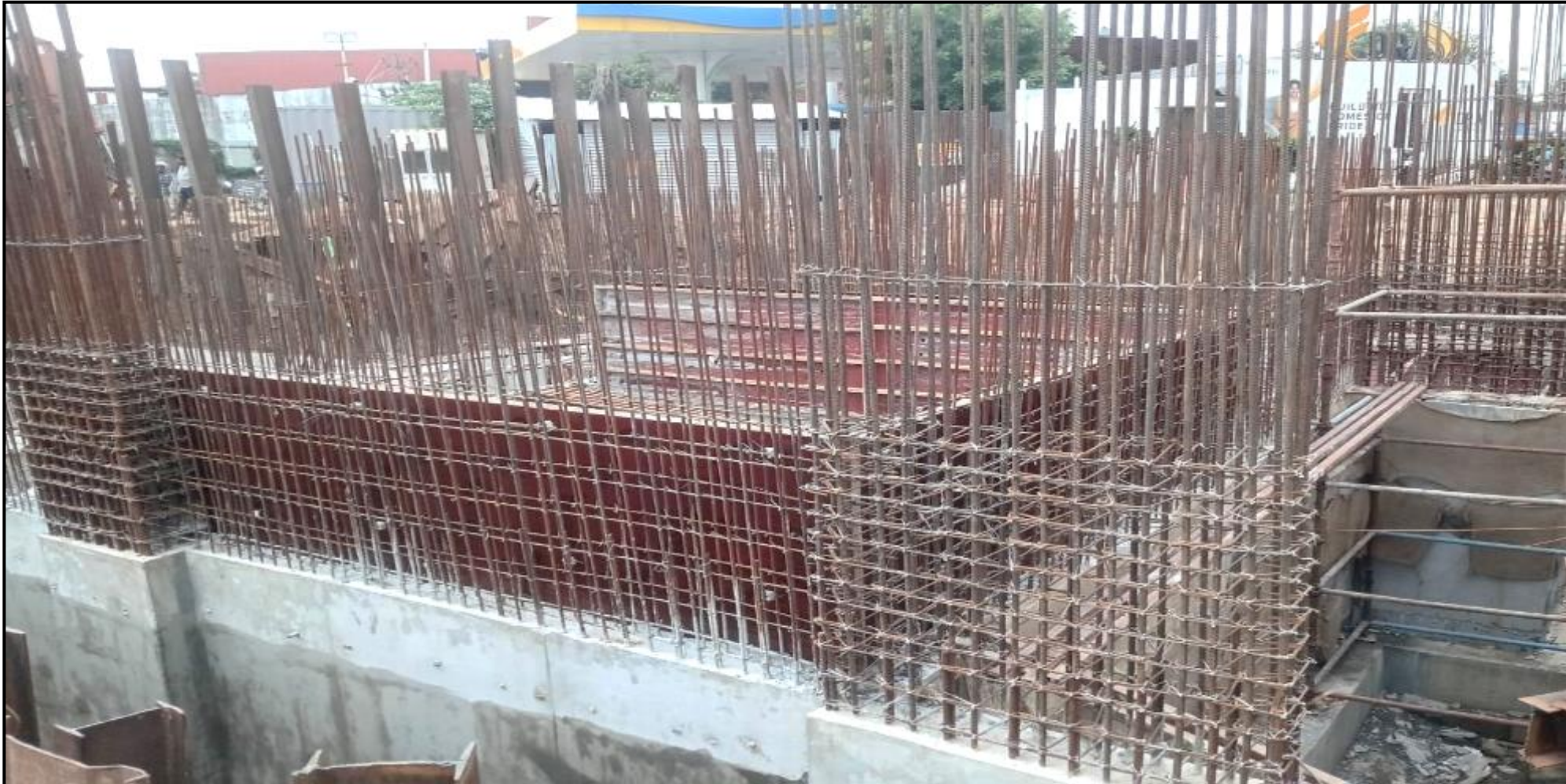
UG Sump – Pour 2 2 nd lift wall reinforcement work in progress
