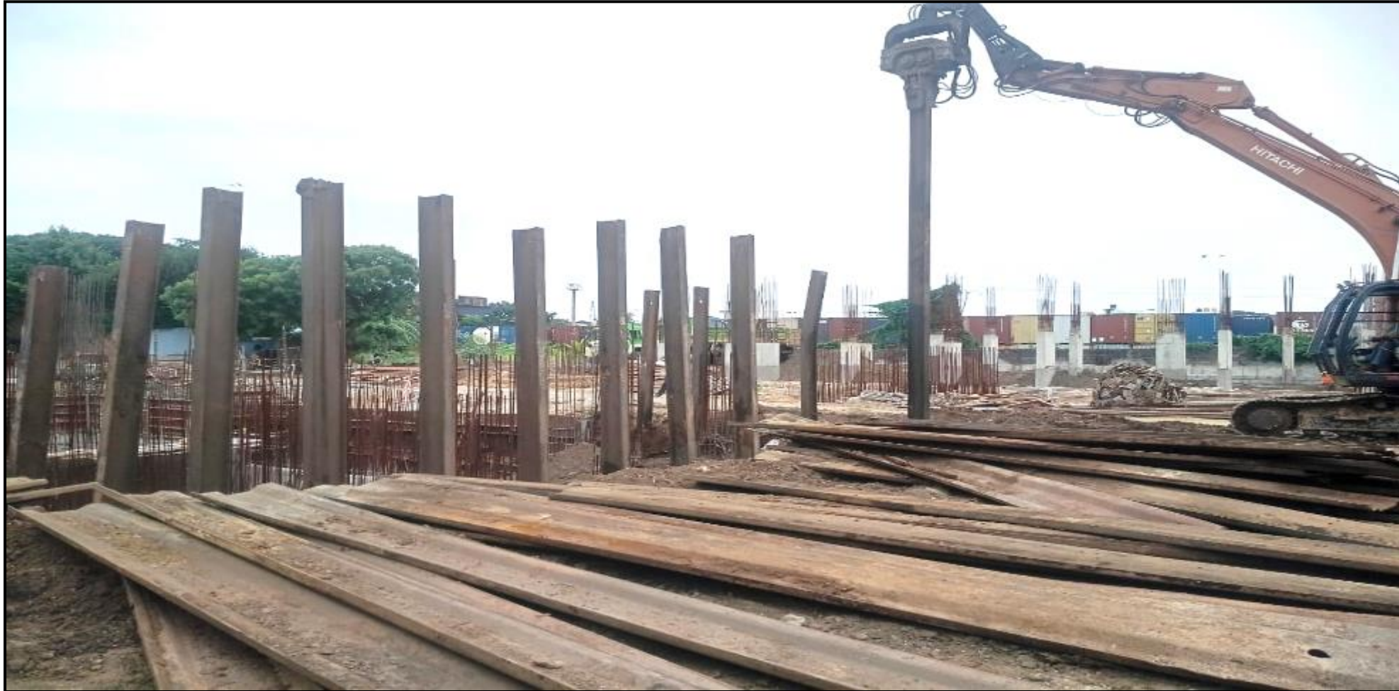
UG Sump – Shoring removing work in progress
