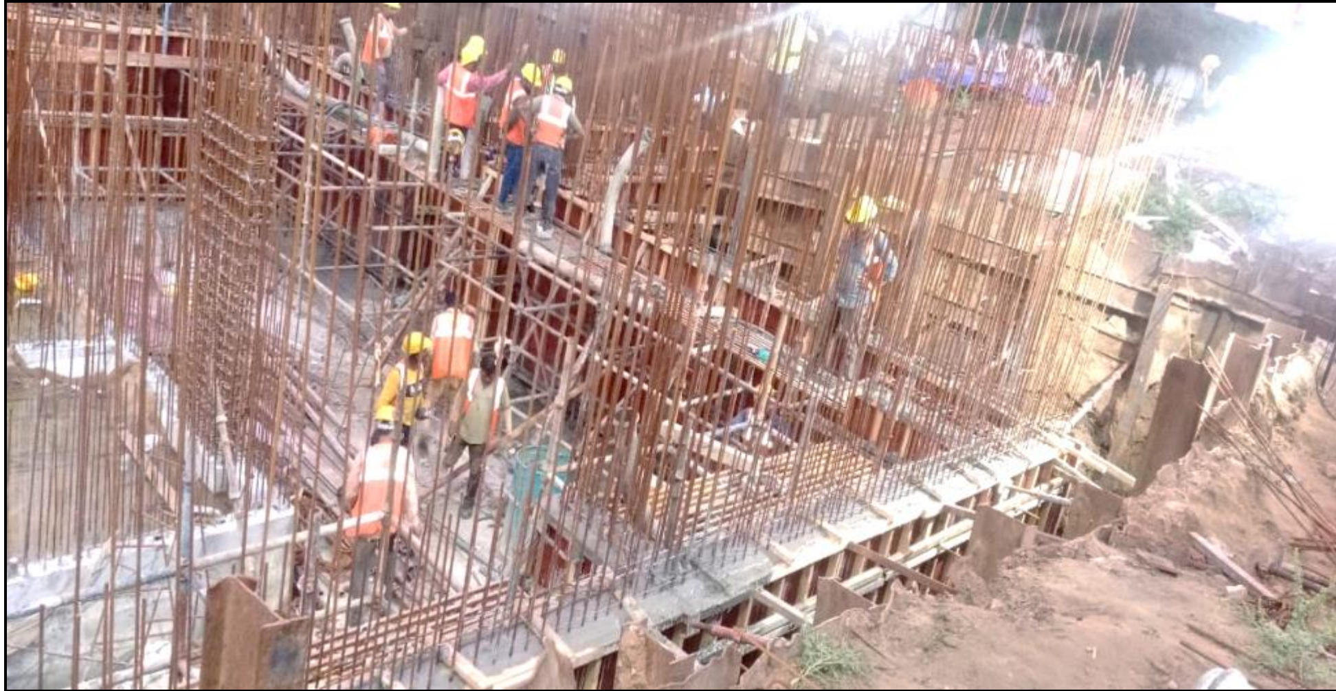
UG Sump Pour 1 – 1 st lift Wall concrete completed
