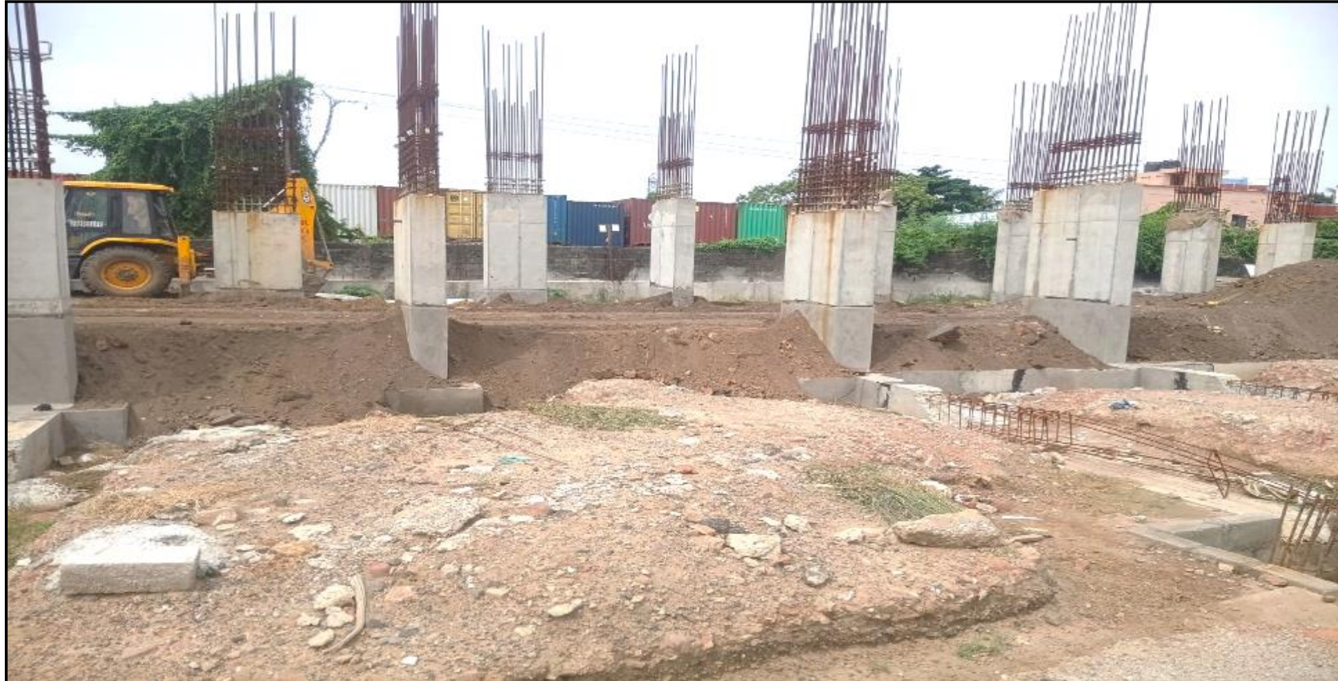
Main building – Basement back filling completed
