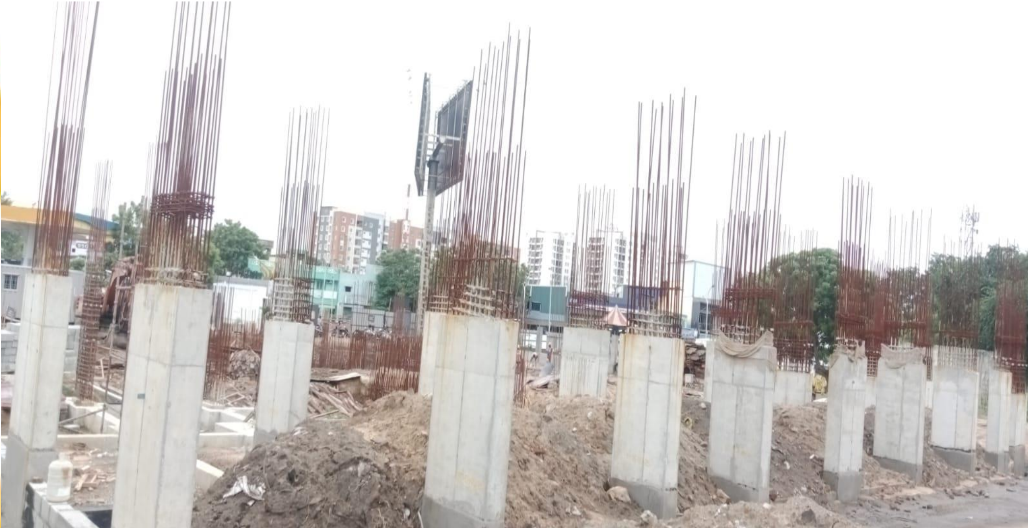
Stilt Floor Column Work in Progress
