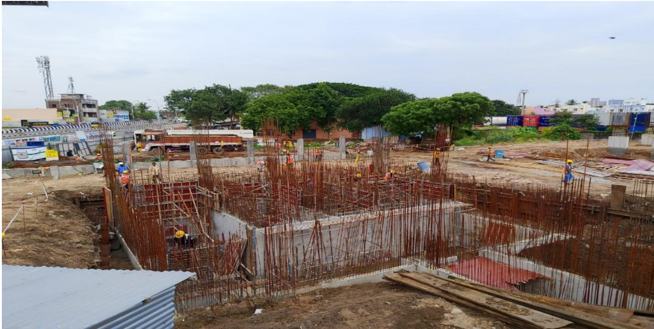
STP – Wall reinforcement work in progress
