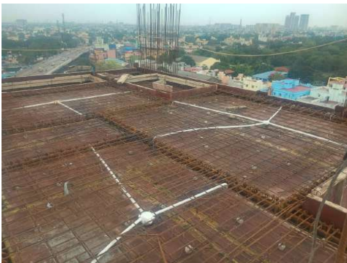
Shuttering - Slab Side
