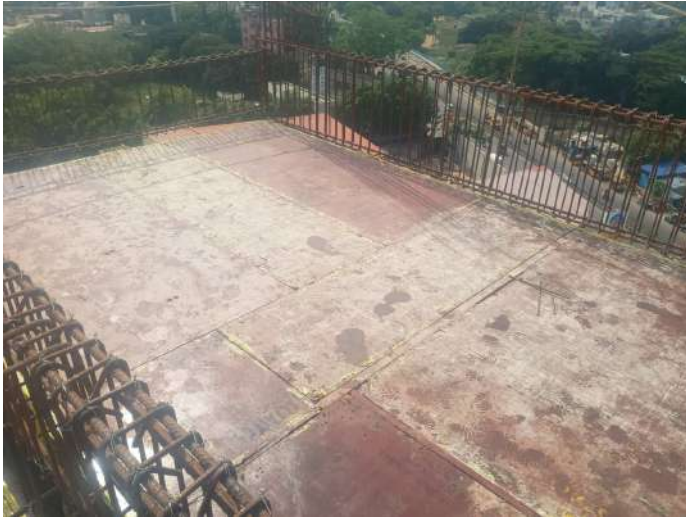
Shuttering -Slab & Beam
