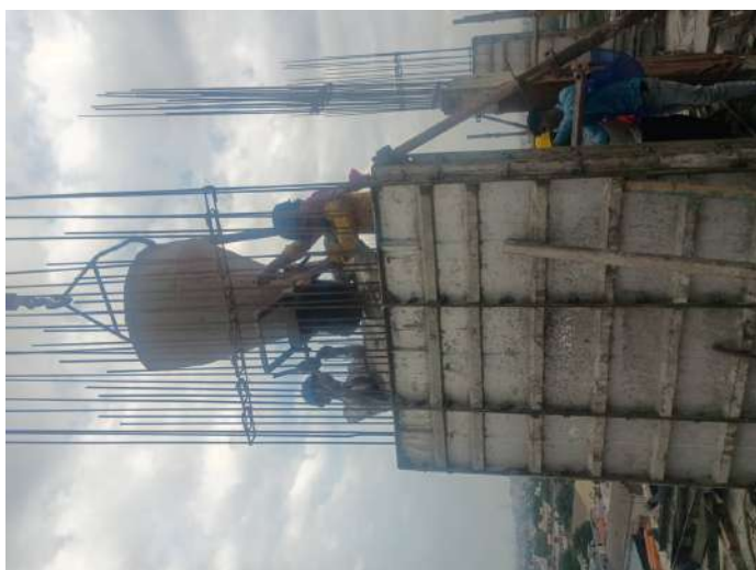
Concreting-Column
