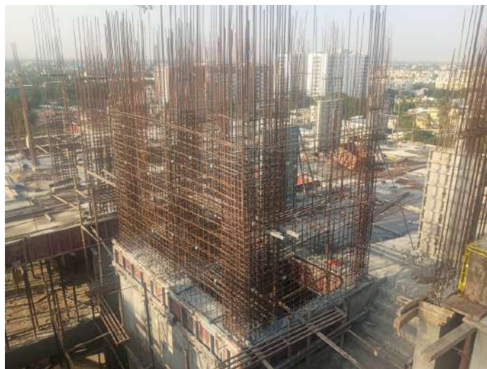
Reinforcement-Column
