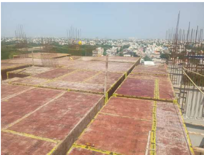
Shuttering -Slab & Beam
