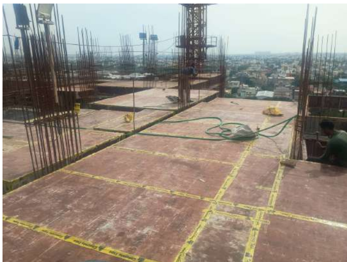
Shuttering -Slab & Beam
