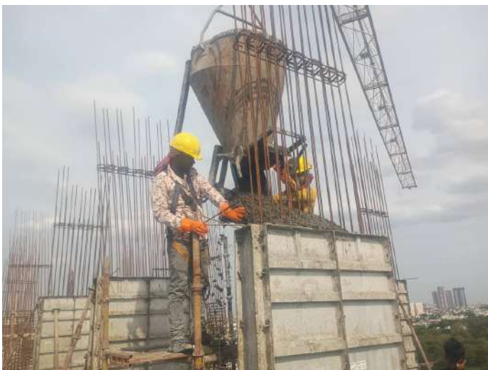
Concreting-Column
