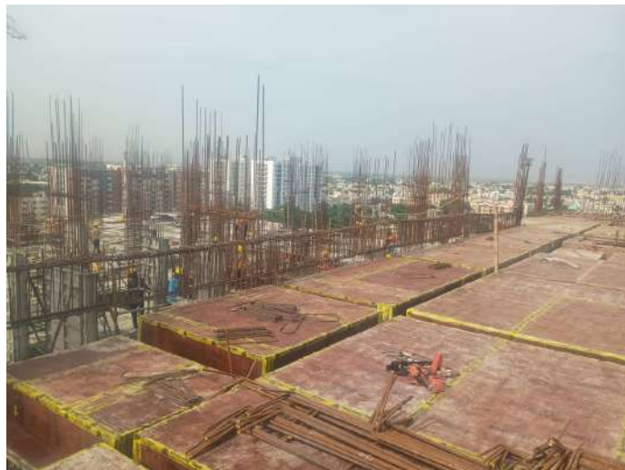
Reinforcement -Slab & Beam
