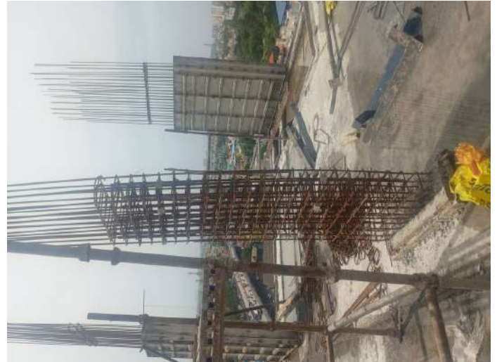
Reinforcement-Column
