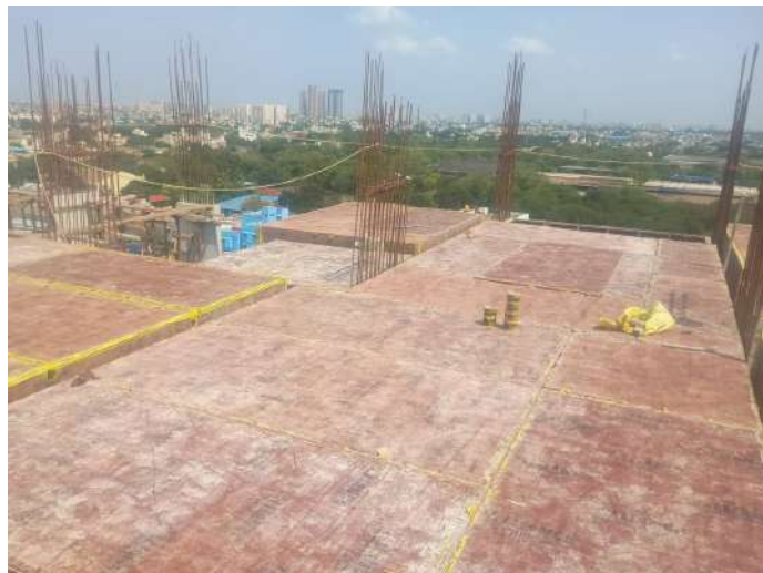
Shuttering -Slab & Beam
