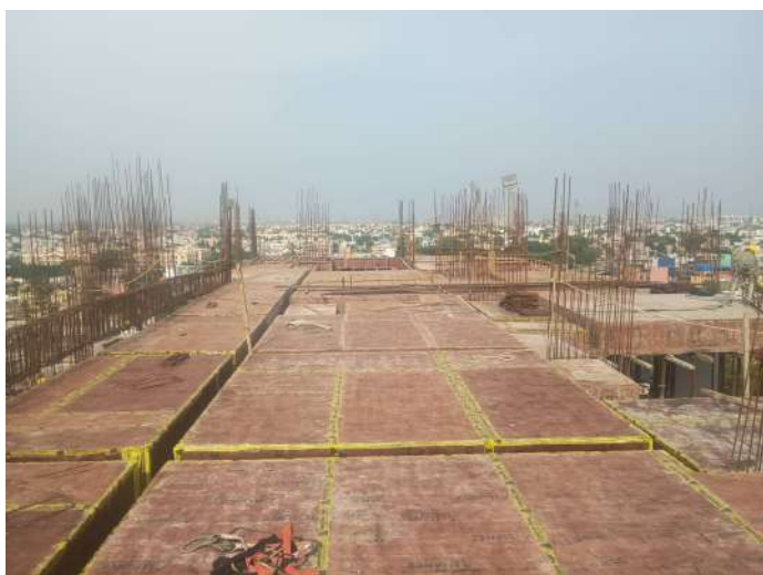
Shuttering -Slab & Beam
