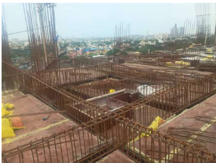
Reinforcement -Slab & Beam
