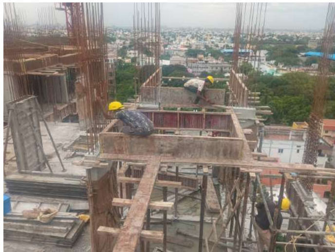
Shuttering -Slab & Beam
