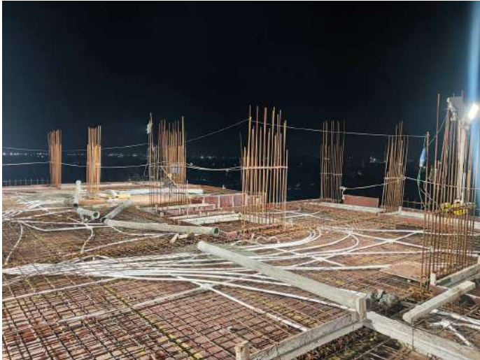
Electrical Works -Slab & Beam
