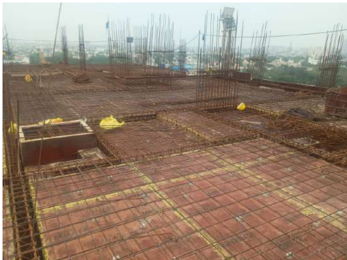
Reinforcement -Slab & Beam
