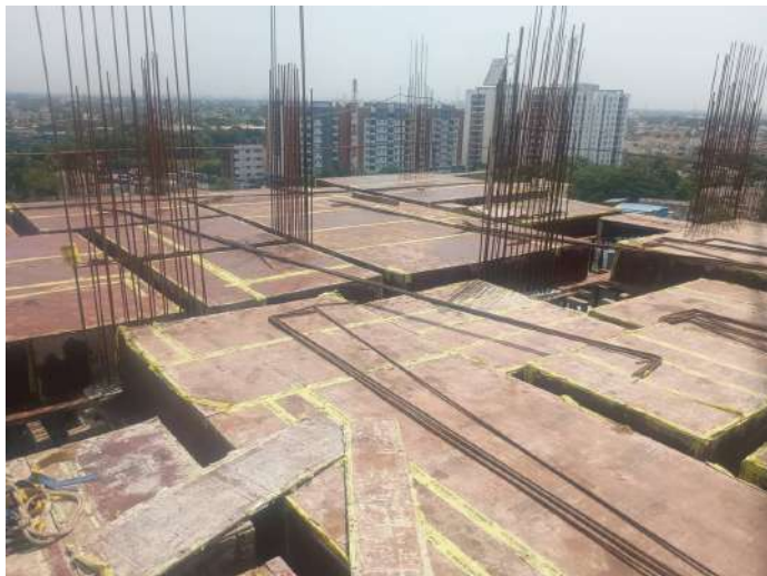
Shuttering -Slab & Beam
