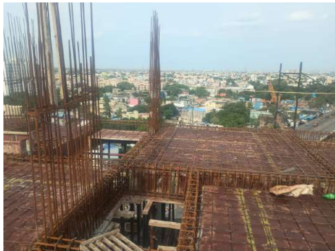
Reinforcement - Slab & Beam
