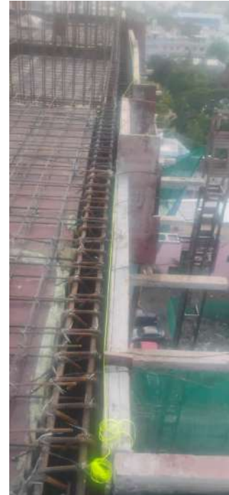
Shuttering - Slab Side
