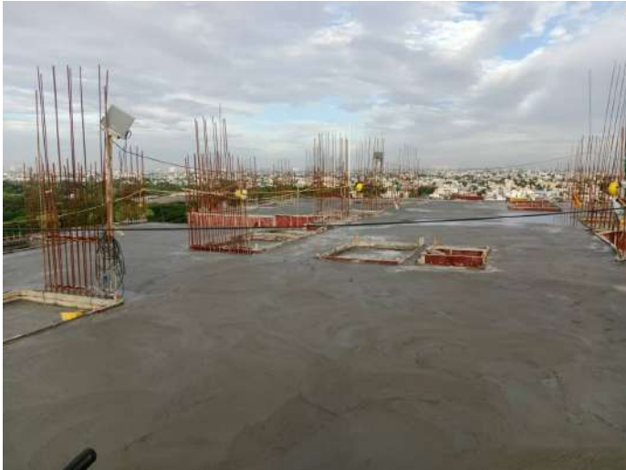
Concreting -Slab & Beam
