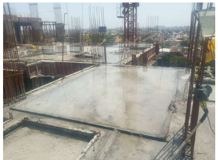
Concreting -Slab & Beam
