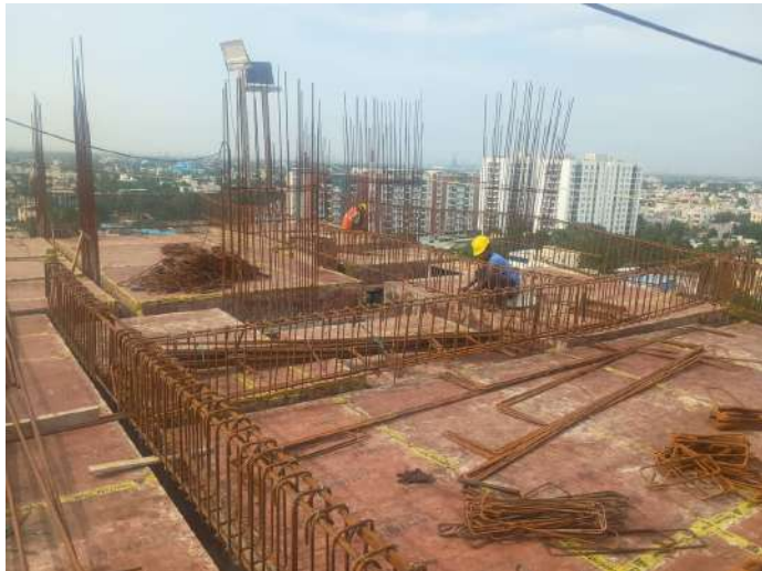
Reinforcement -Slab & Beam
