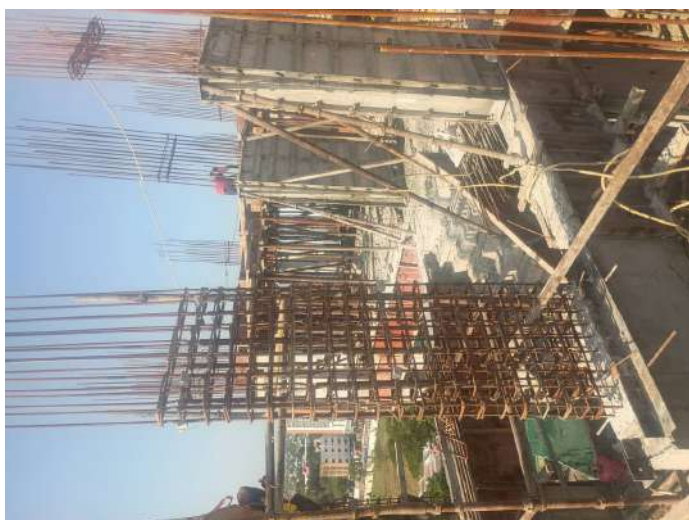
Reinforcement-Column
