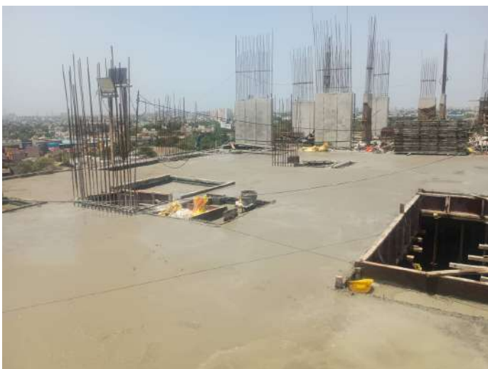
Concreting -Slab & Beam
