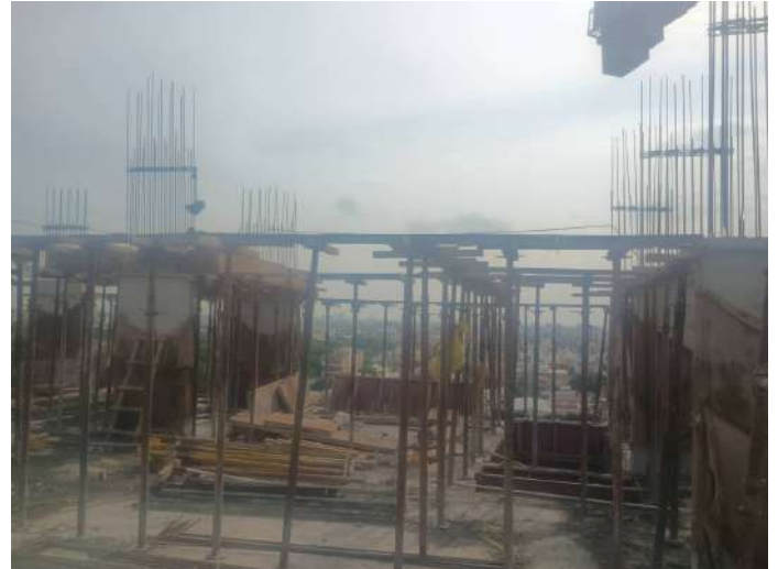
Shuttering -Slab & Beam
