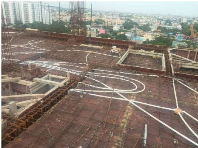
Reinforcement -Slab & Beam
