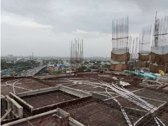
Electrical Works -Slab & Beam
