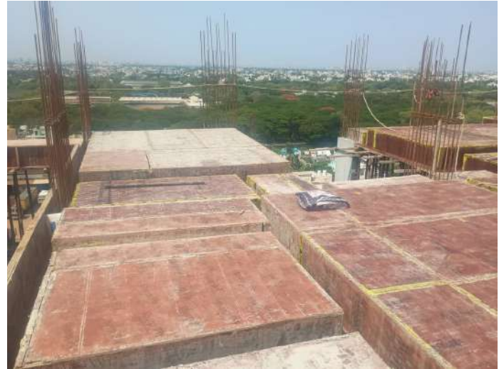
Shuttering -Slab & Beam
