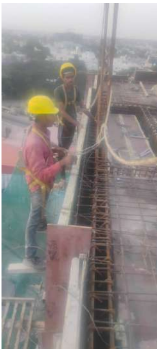
Shuttering - Slab Side
