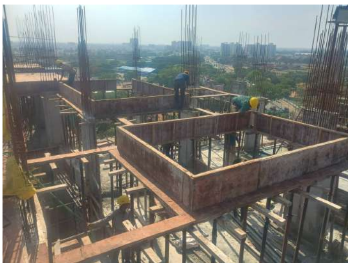
Shuttering -Slab & Beam
