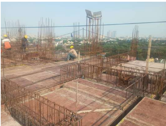
Shuttering -Slab & Beam
