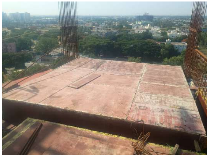
Shuttering -Slab & Beam
