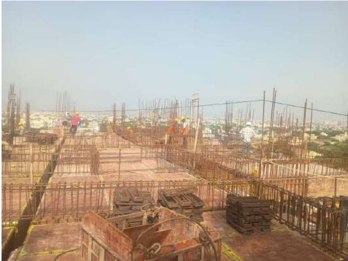
Reinforcement -Slab & Beam
