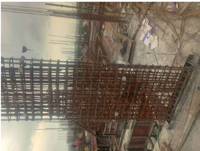
Reinforcement-Column
