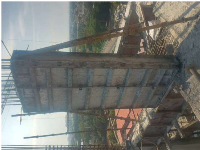
Concreting-Column
