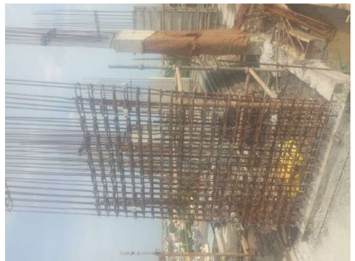
Reinforcement-Column
