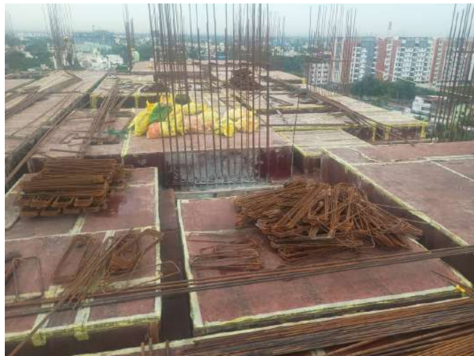
Reinforcement -Slab & Beam
