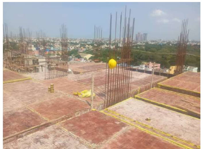
Shuttering -Slab & Beam
