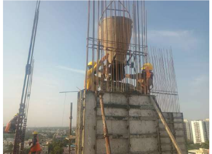
Concreting-Column
