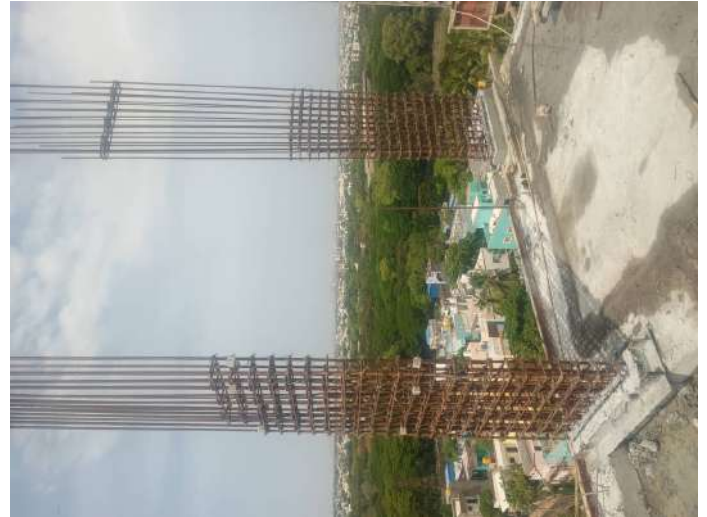
Reinforcement-Column
