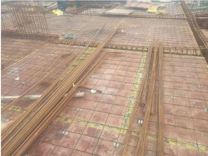
Reinforcement -Slab & Beam
