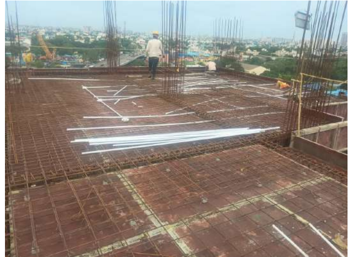
Reinforcement -Slab & Beam
