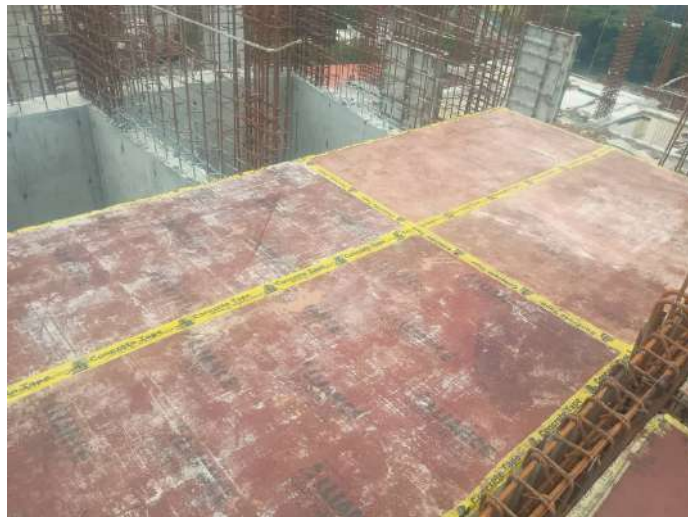
Shuttering -Slab & Beam
