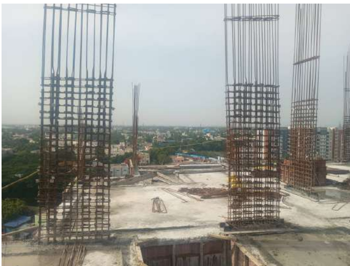
Reinforcement-Column
