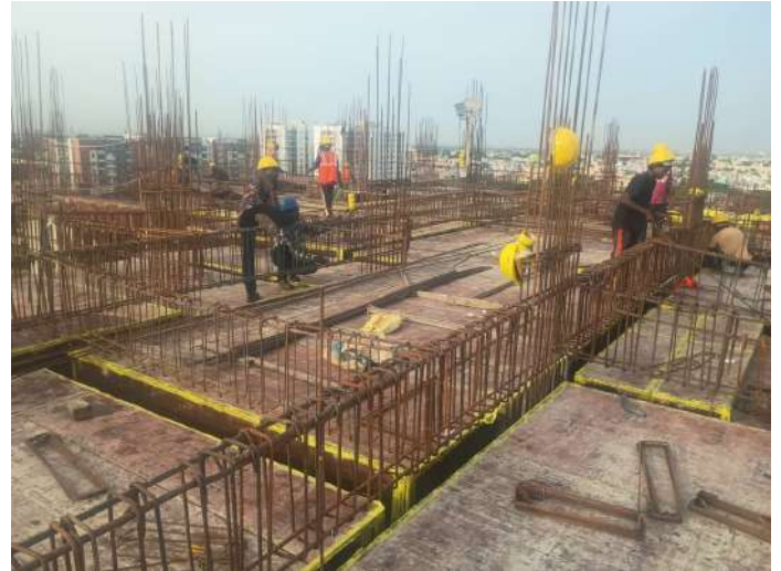
Reinforcement -Slab & Beam
