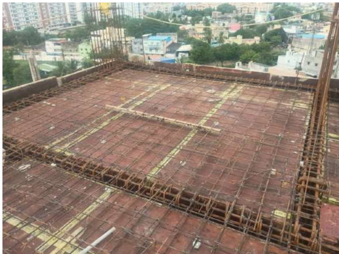
Reinforcement -Slab & Beam
