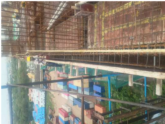
Shuttering - Slab Side
