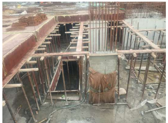
Shuttering -Slab & Beam
