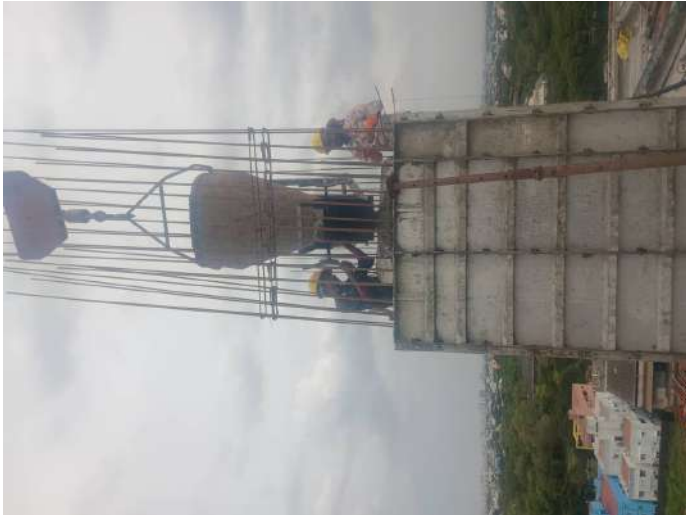
Concreting-Column
