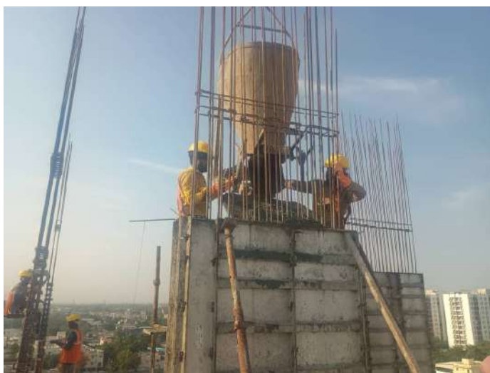
Concreting-Column
