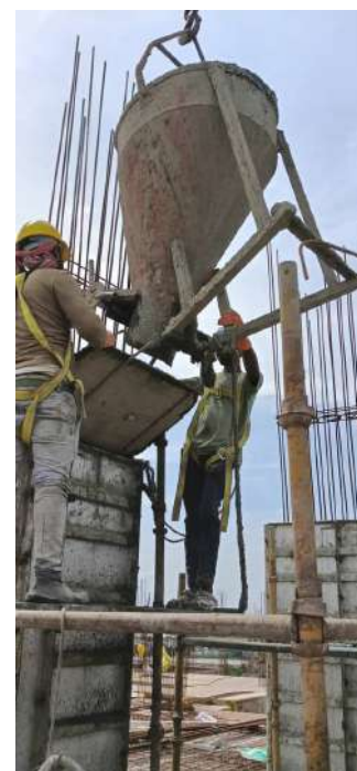
Concreting-Column
