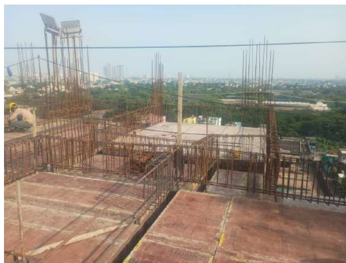
Reinforcement -Slab & Beam
