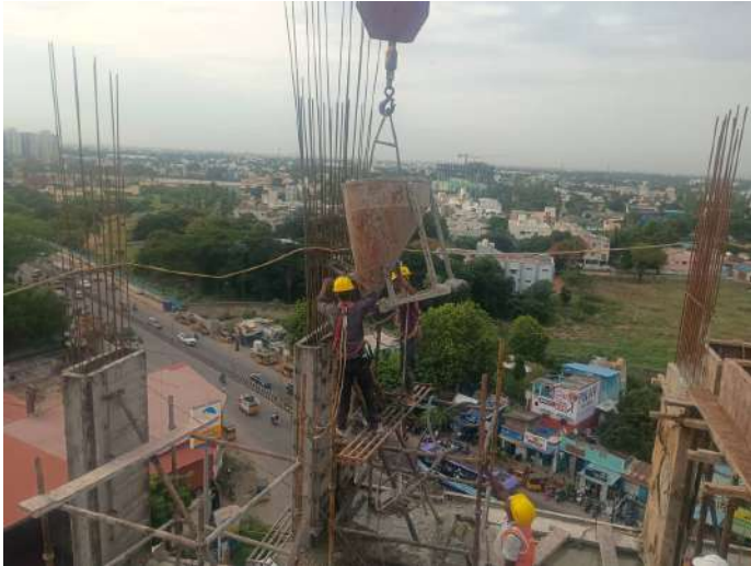
Concreting-Column
