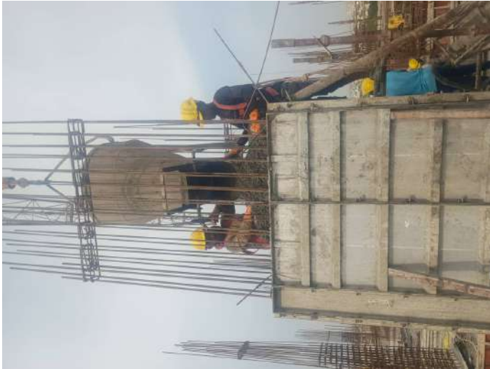
Concreting-Column
