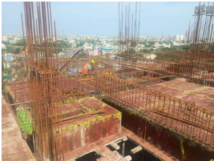
Reinforcement -Slab & Beam
