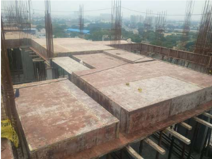
Shuttering -Slab & Beam
