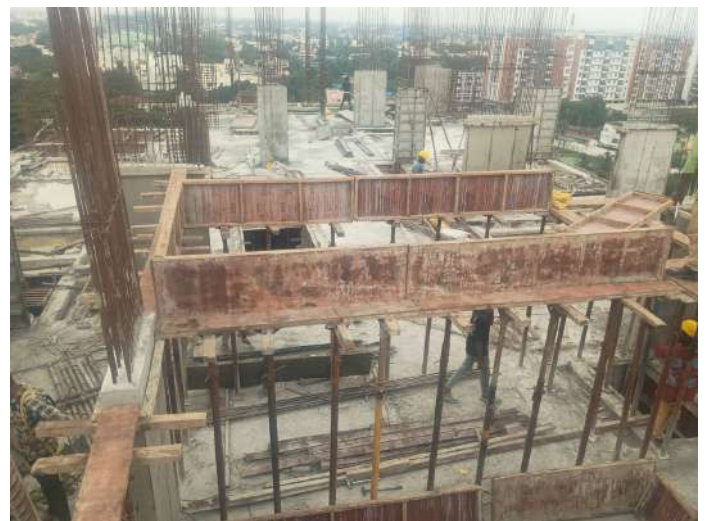
Shuttering -Slab & Beam
