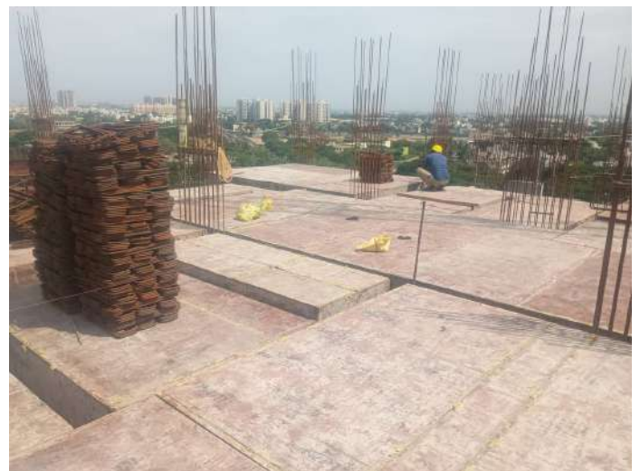
Shuttering -Slab & Beam
