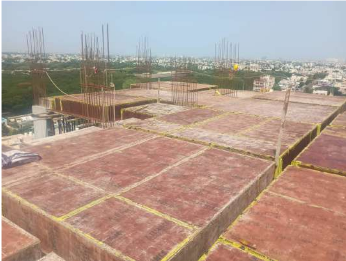
Shuttering -Slab & Beam
