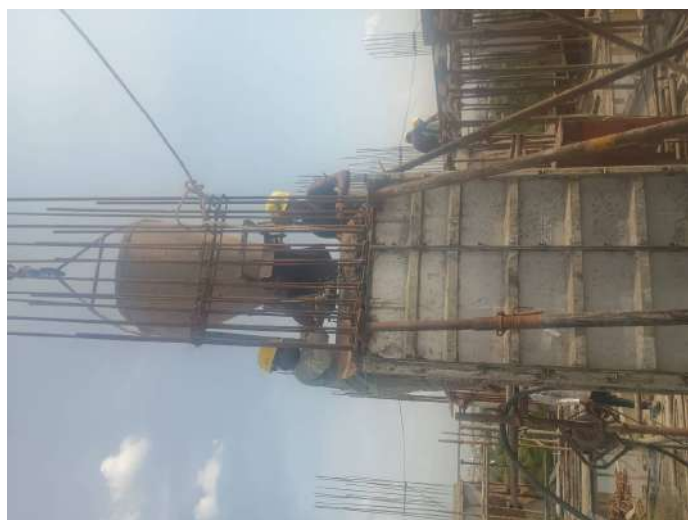
Concreting-Column
