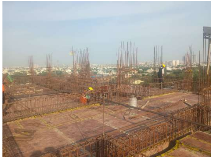
Reinforcement -Slab & Beam
