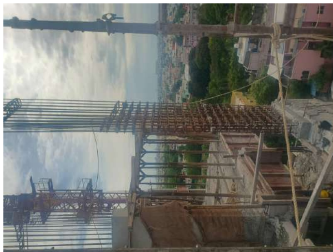
Reinforcement-Column
