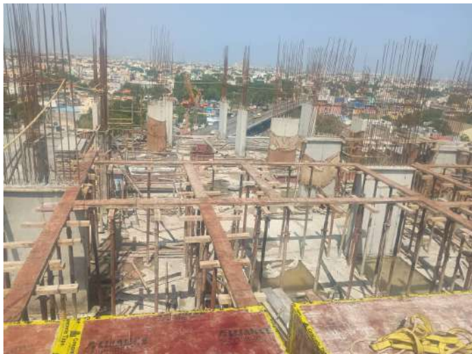
Shuttering -Slab & Beam
