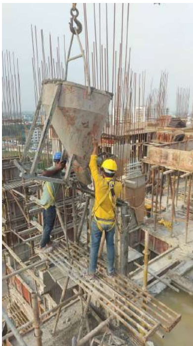
Concreting-Column
