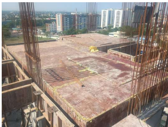
Shuttering -Slab & Beam
