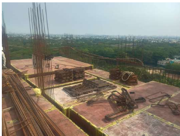
Shuttering -Slab & Beam
