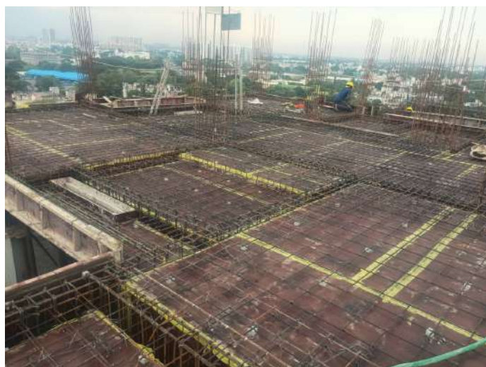
Reinforcement -Slab & Beam
