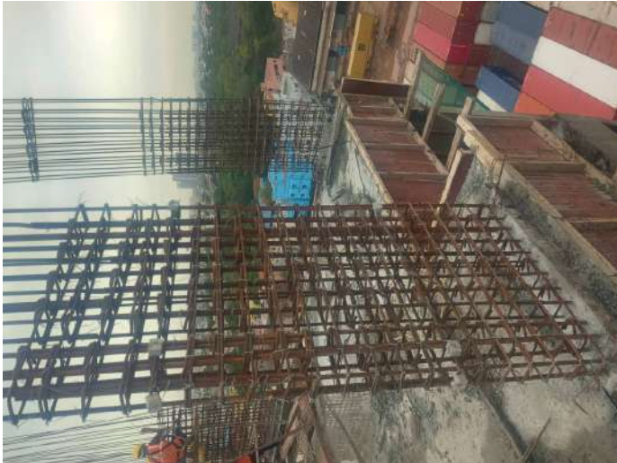
Reinforcement-Column
