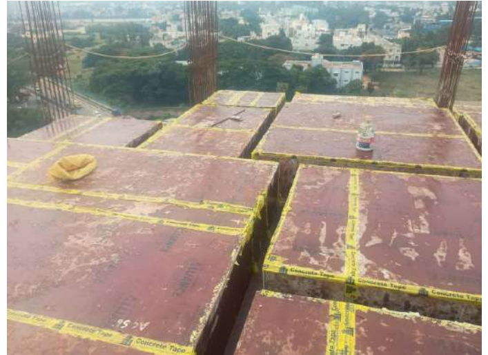
Shuttering -Slab & Beam
