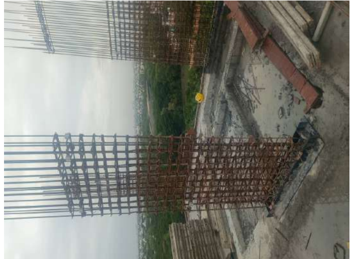
Reinforcement-Column
