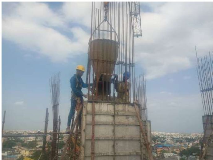
Concreting-Column
