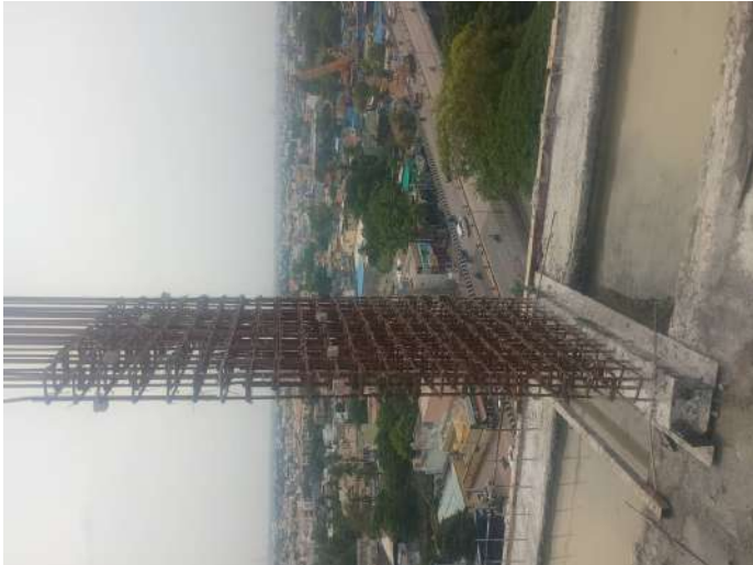
Reinforcement-Column
