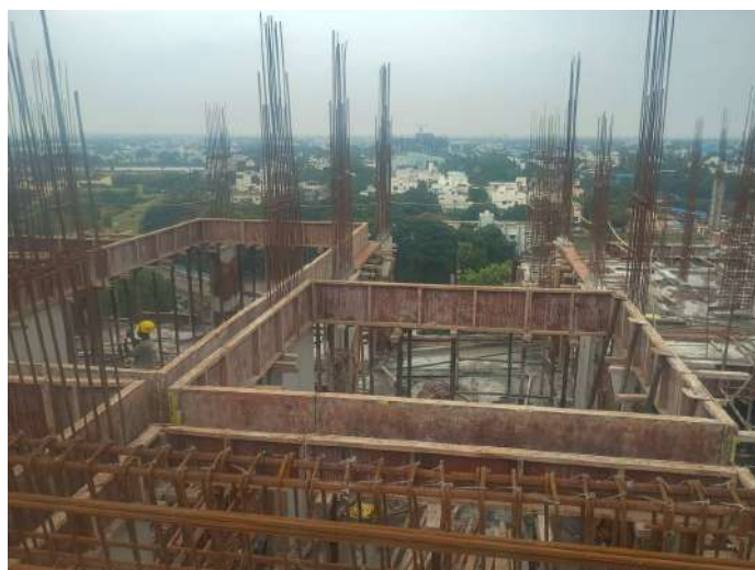
Shuttering -Slab & Beam
