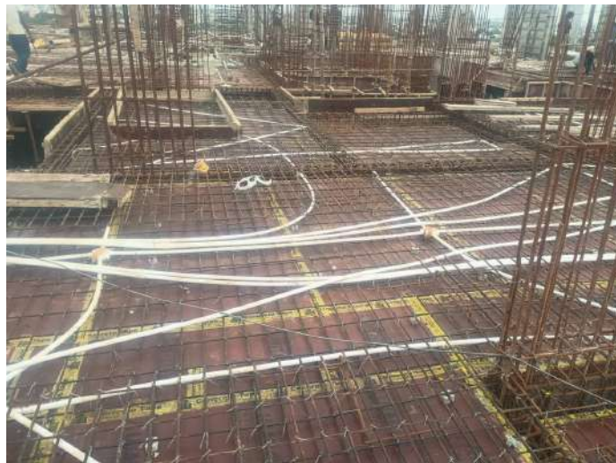
Reinforcement -Slab & Beam
