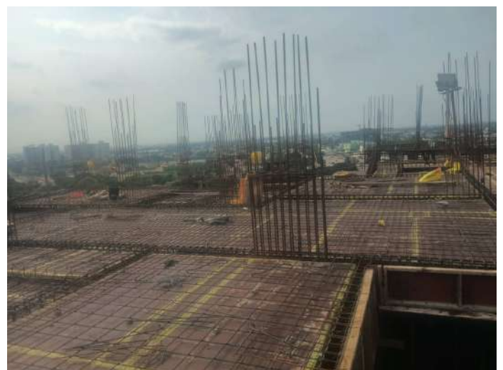
Reinforcement - Slab & Beam
