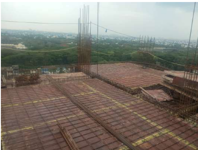
Reinforcement -Slab & Beam
