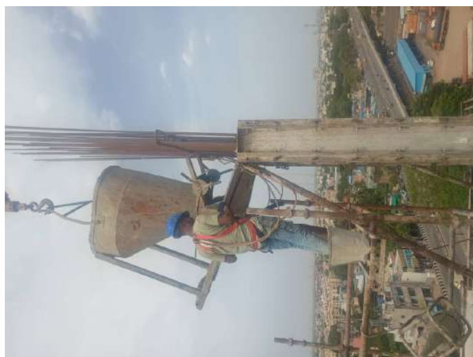
Concreting-Column
