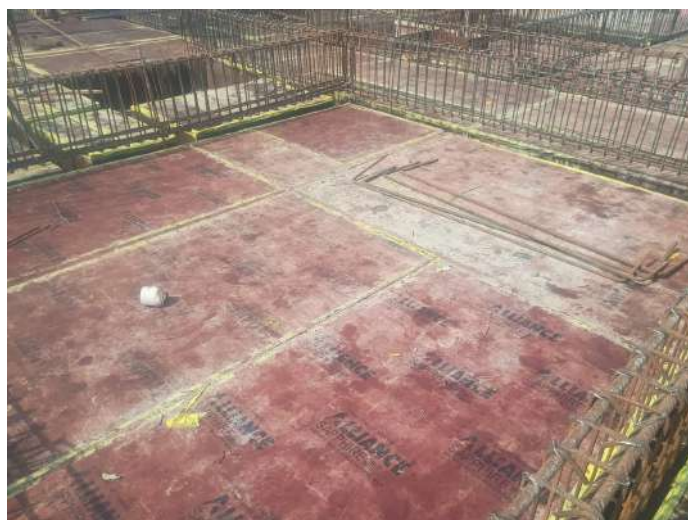
Shuttering -Slab & Beam
