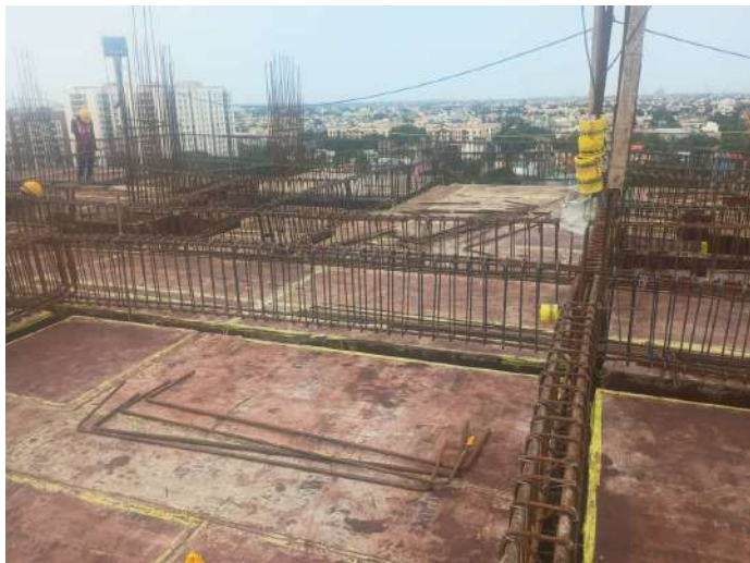
Reinforcement -Slab & Beam
