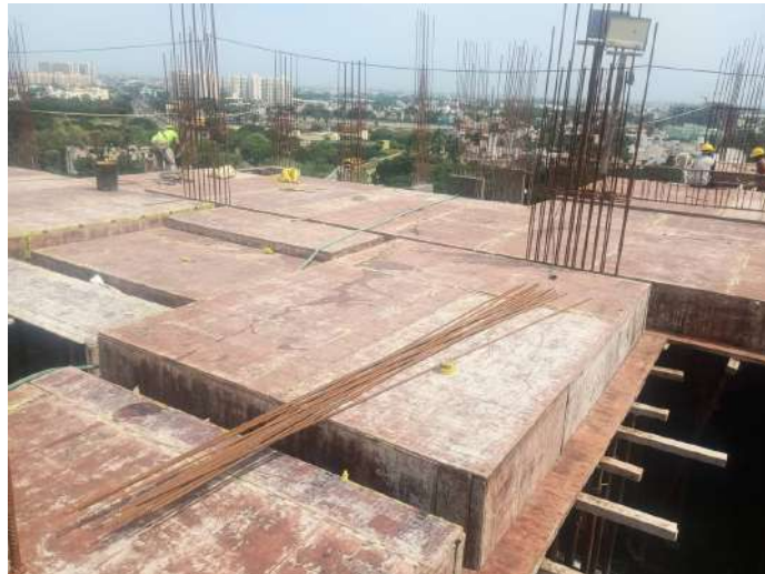
Shuttering -Slab & Beam
