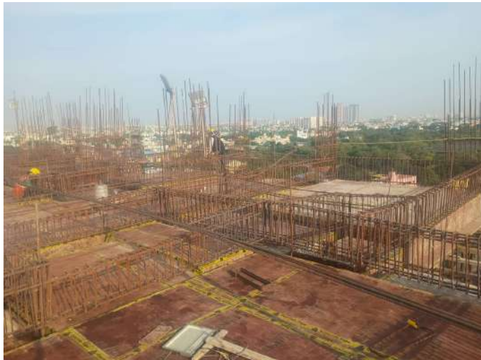
Reinforcement -Slab & Beam
