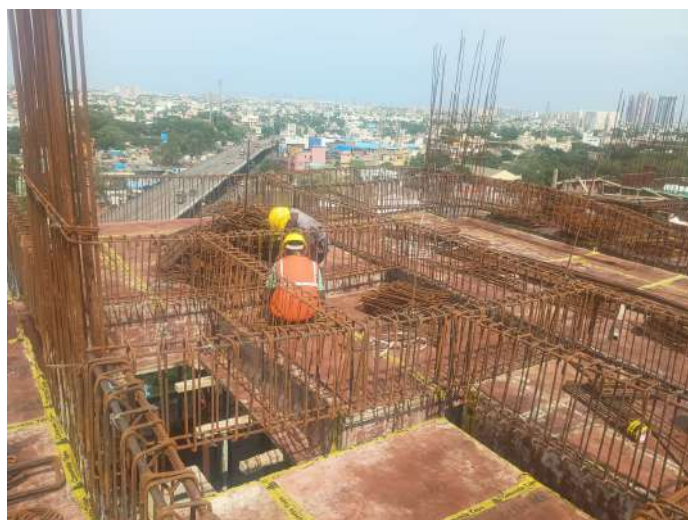
Reinforcement -Slab & Beam
