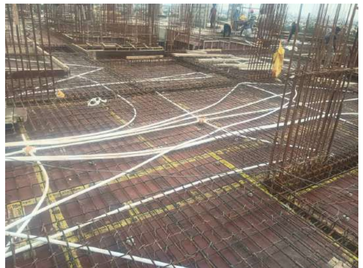
Reinforcement -Slab & Beam
