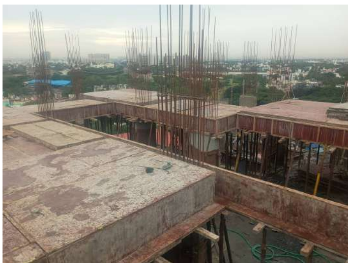
Shuttering -Slab & Beam
