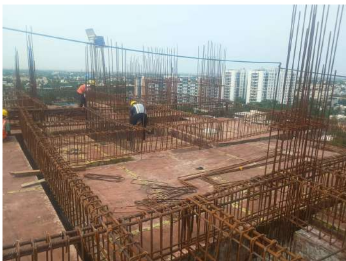
Reinforcement - Slab & Beam
