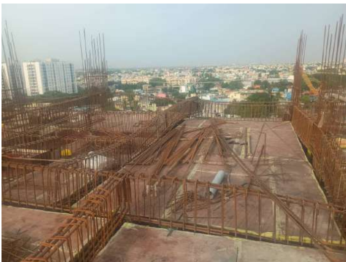
Reinforcement -Slab & Beam
