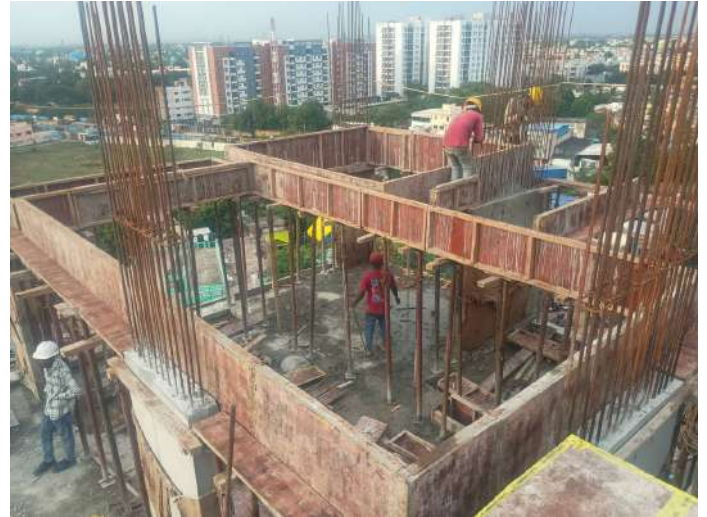
Shuttering -Slab & Beam
