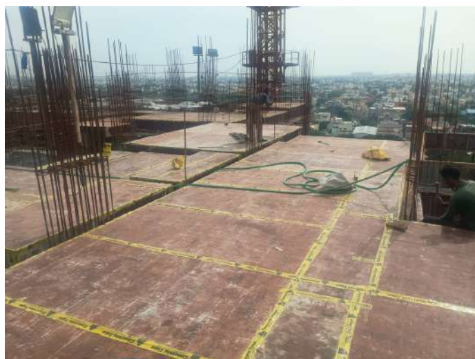
Shuttering - Slab & Beam
