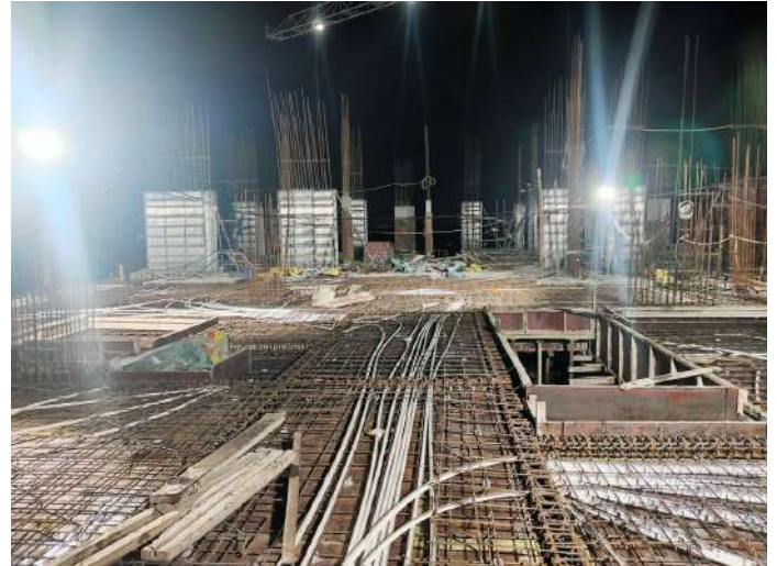
Electrical Works -Slab & Beam
