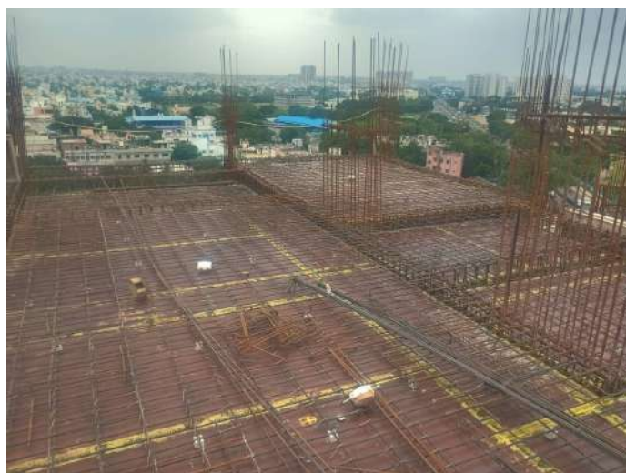
Reinforcement -Slab & Beam
