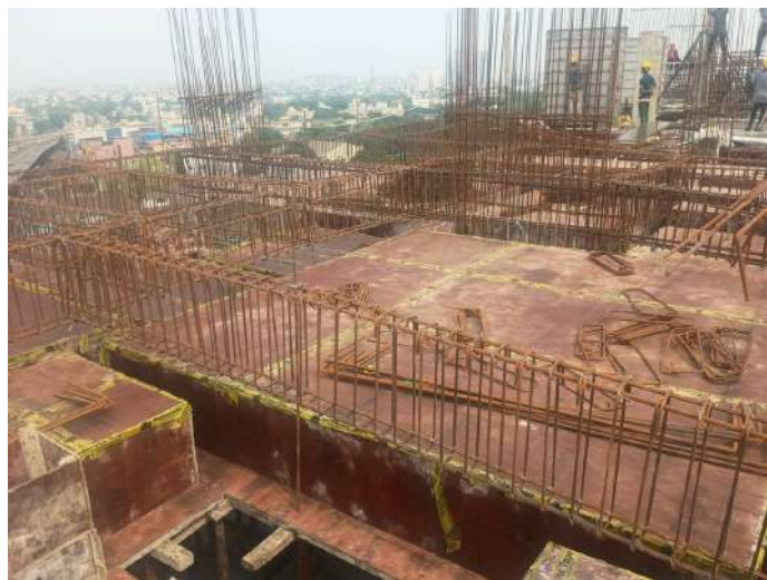
Reinforcement -Slab & Beam
