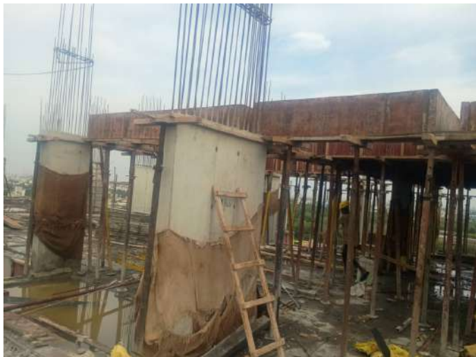
Shuttering -Slab & Beam
