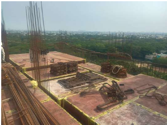
Reinforcement -Slab & Beam
