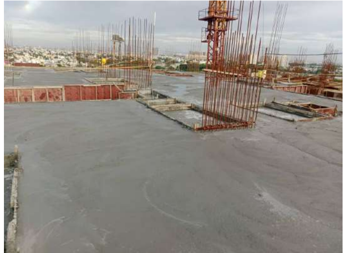
Concreting -Slab & Beam
