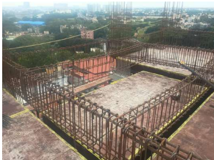
Reinforcement -Slab & Beam
