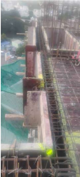
Shuttering - Slab Side
