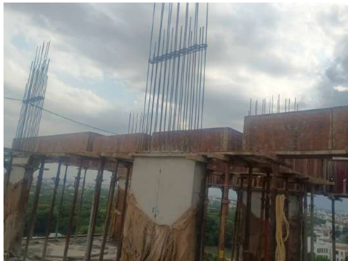
Shuttering -Slab & Beam
