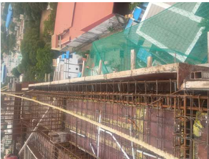
Shuttering - Slab Side
