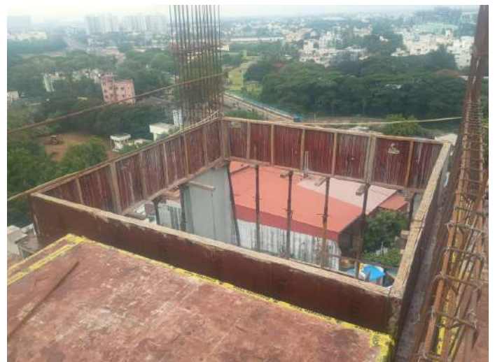
Shuttering -Slab & Beam
