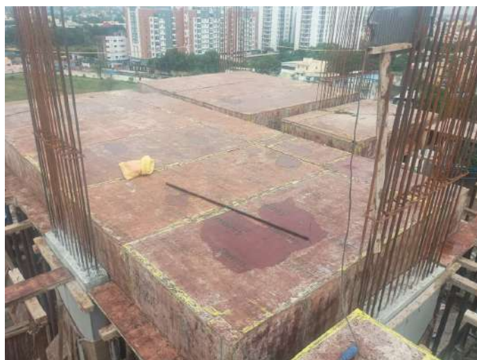
Shuttering -Slab & Beam
