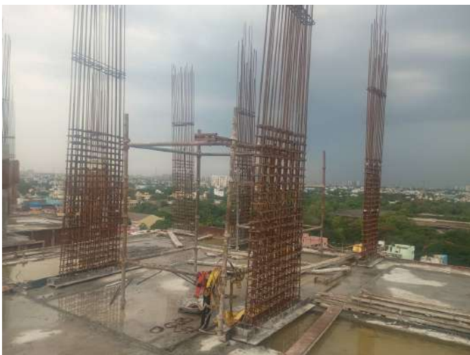
Reinforcement-Column
