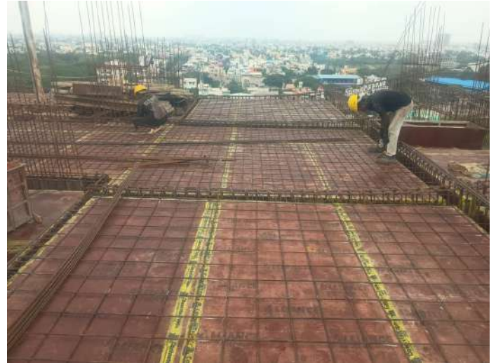
Reinforcement -Slab & Beam
