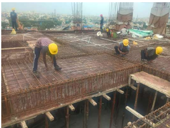
Reinforcement -Slab & Beam
