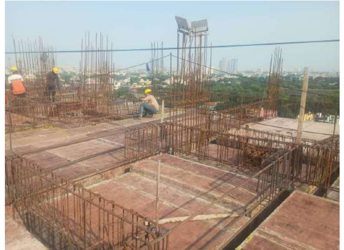
Reinforcement -Slab & Beam
