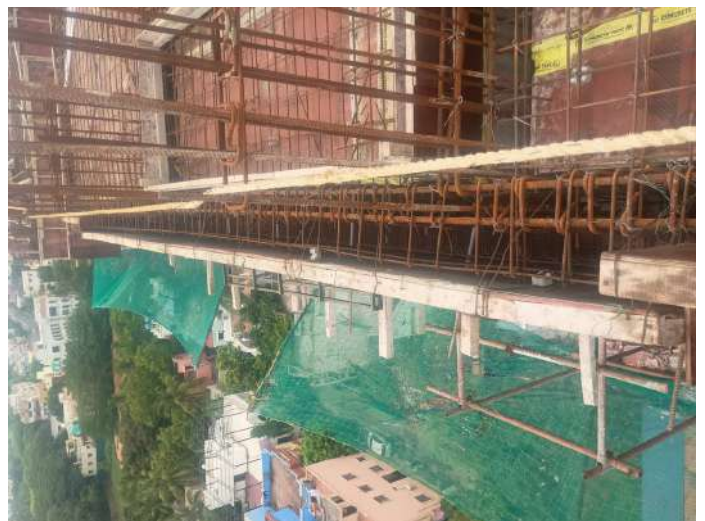
Shuttering - Slab Side
