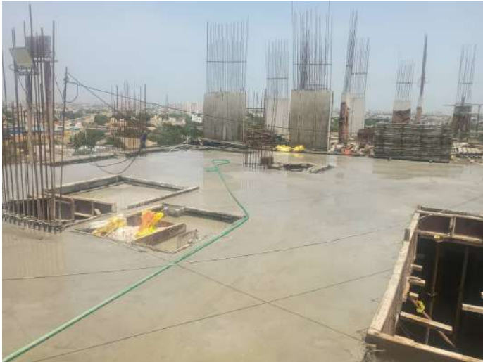
Concreting -Slab & Beam
