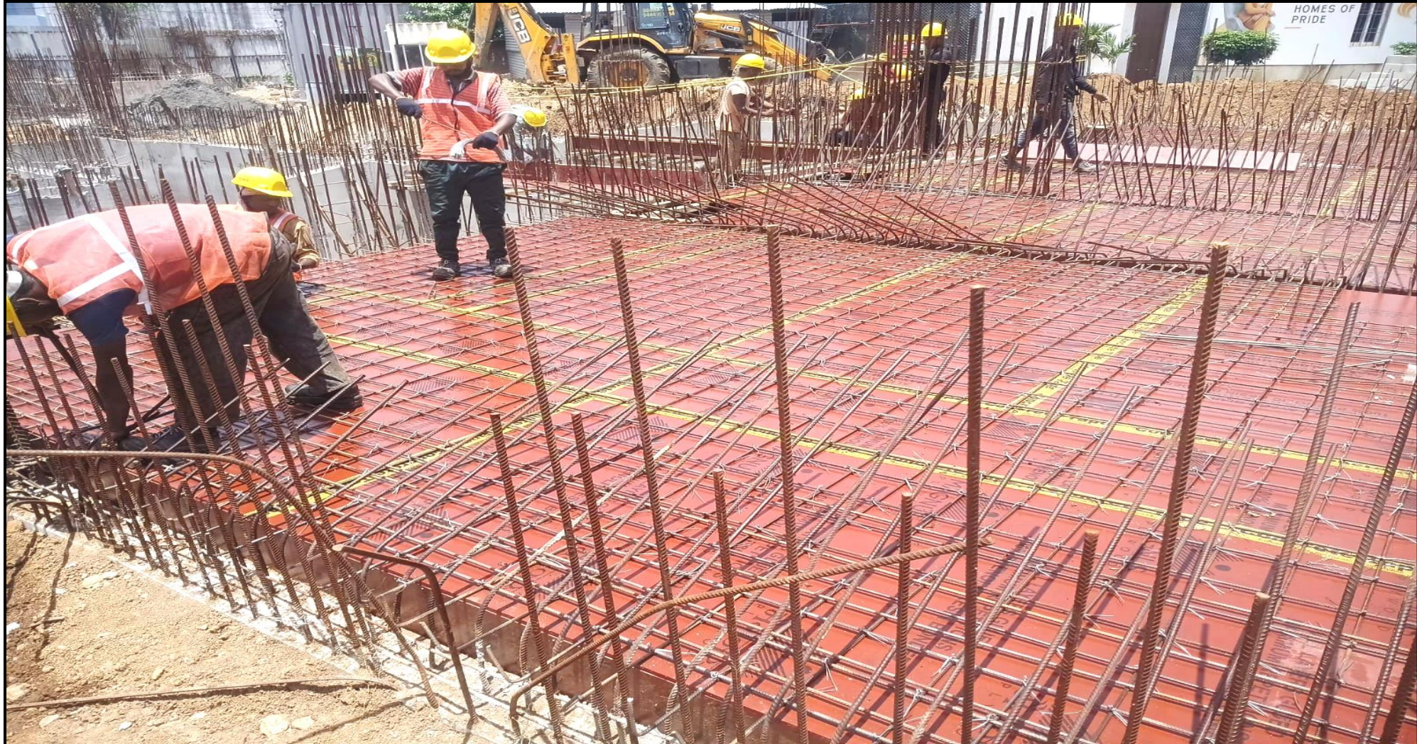
UG Sump – Cover slab reinforcement work in progress
