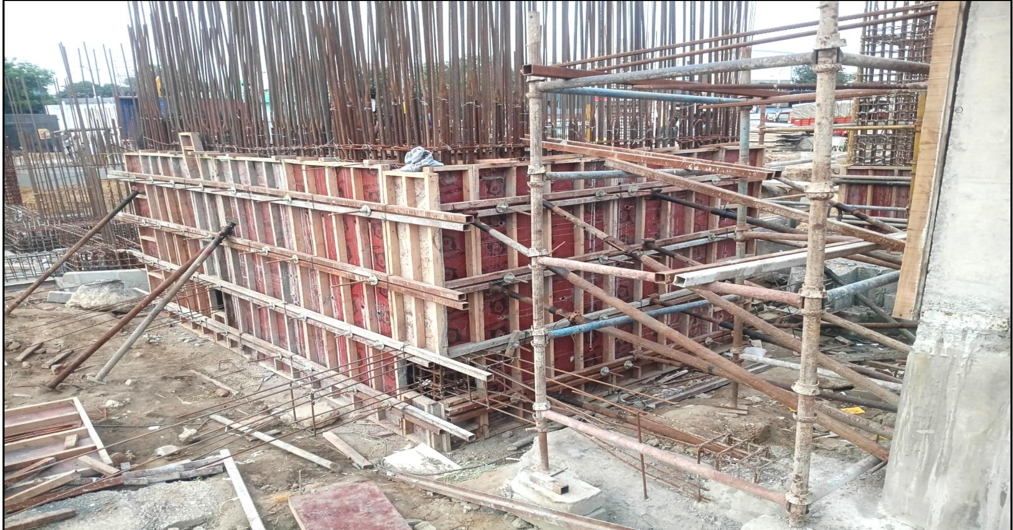
Main building – 1 st Lift core wall shuttering work completed
