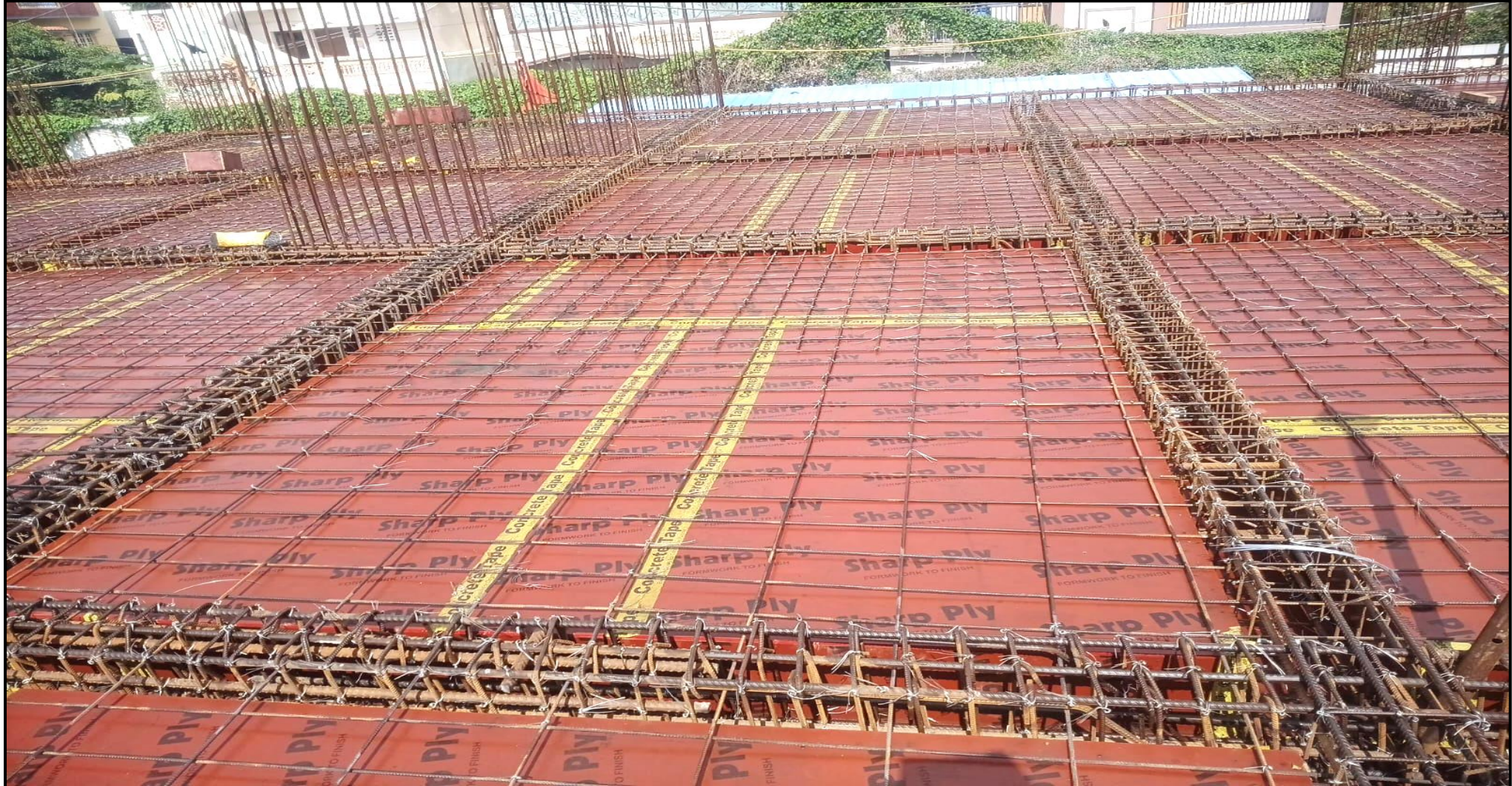
Main building – Pour 1 stilt floor roof slab reinforcement work completed
