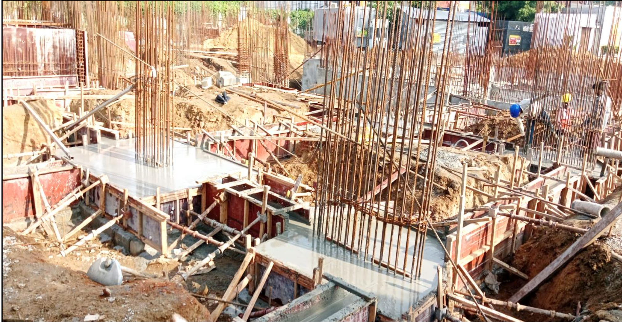
Main building – Pour 2 pile cap concrete completed (47/47 no's )
