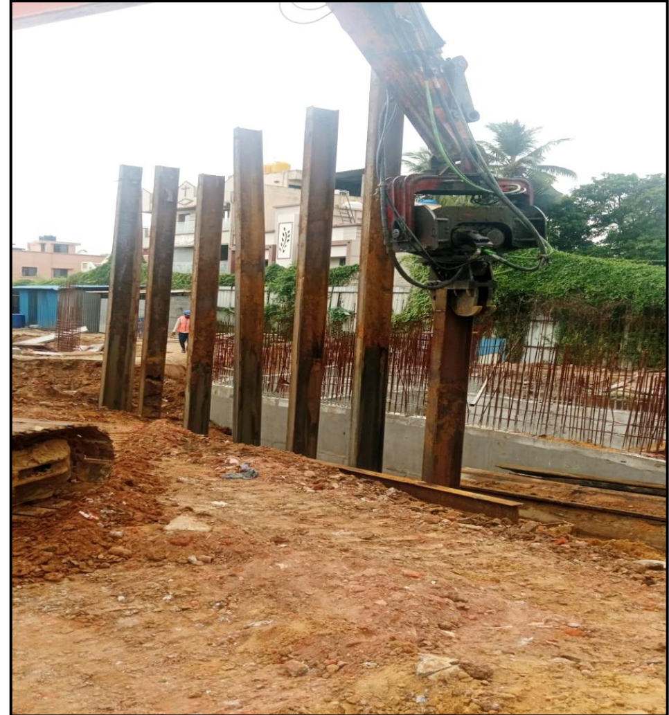
STP – Shoring removal work completed
