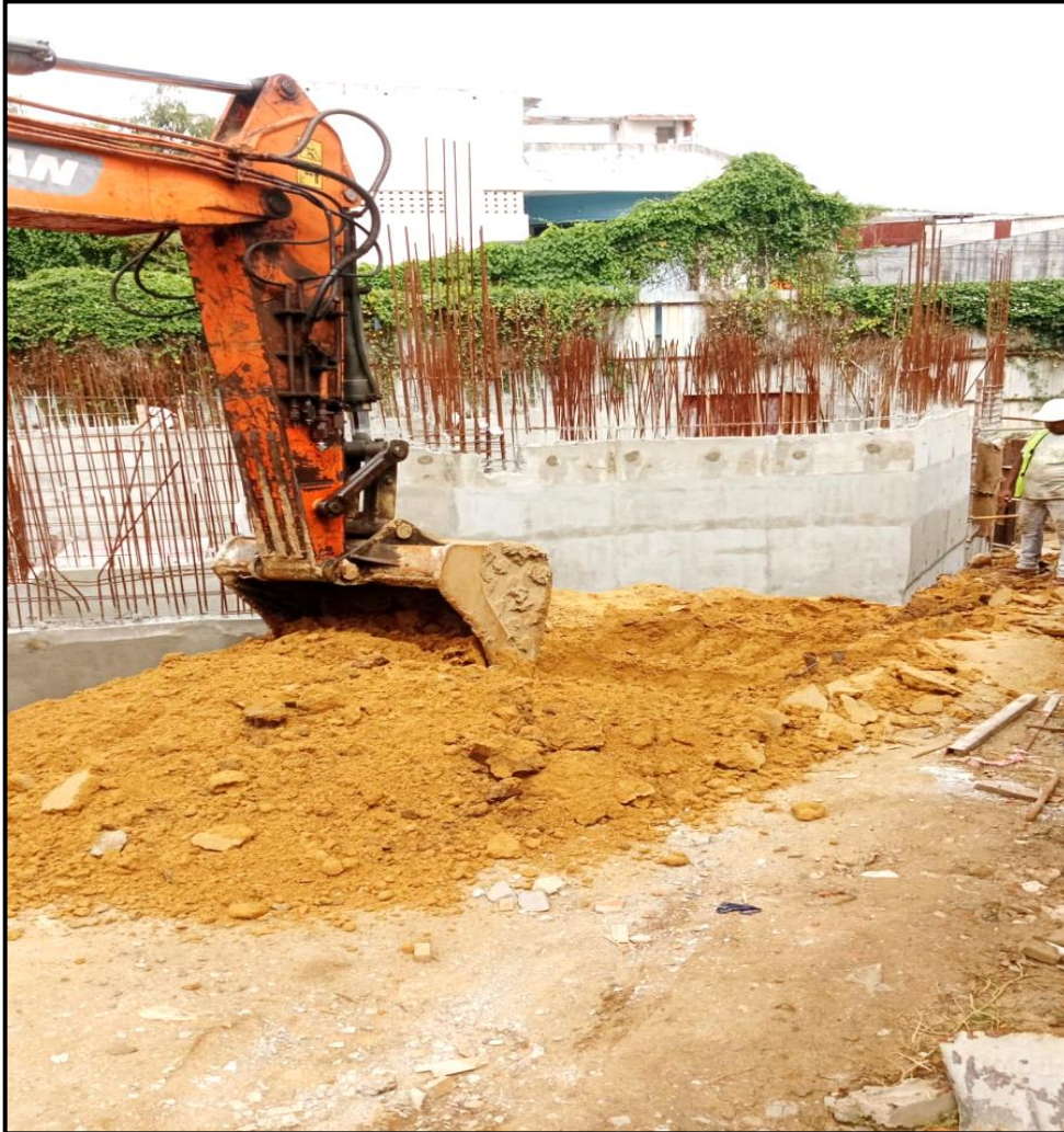
STP – Shoring removal work completed
