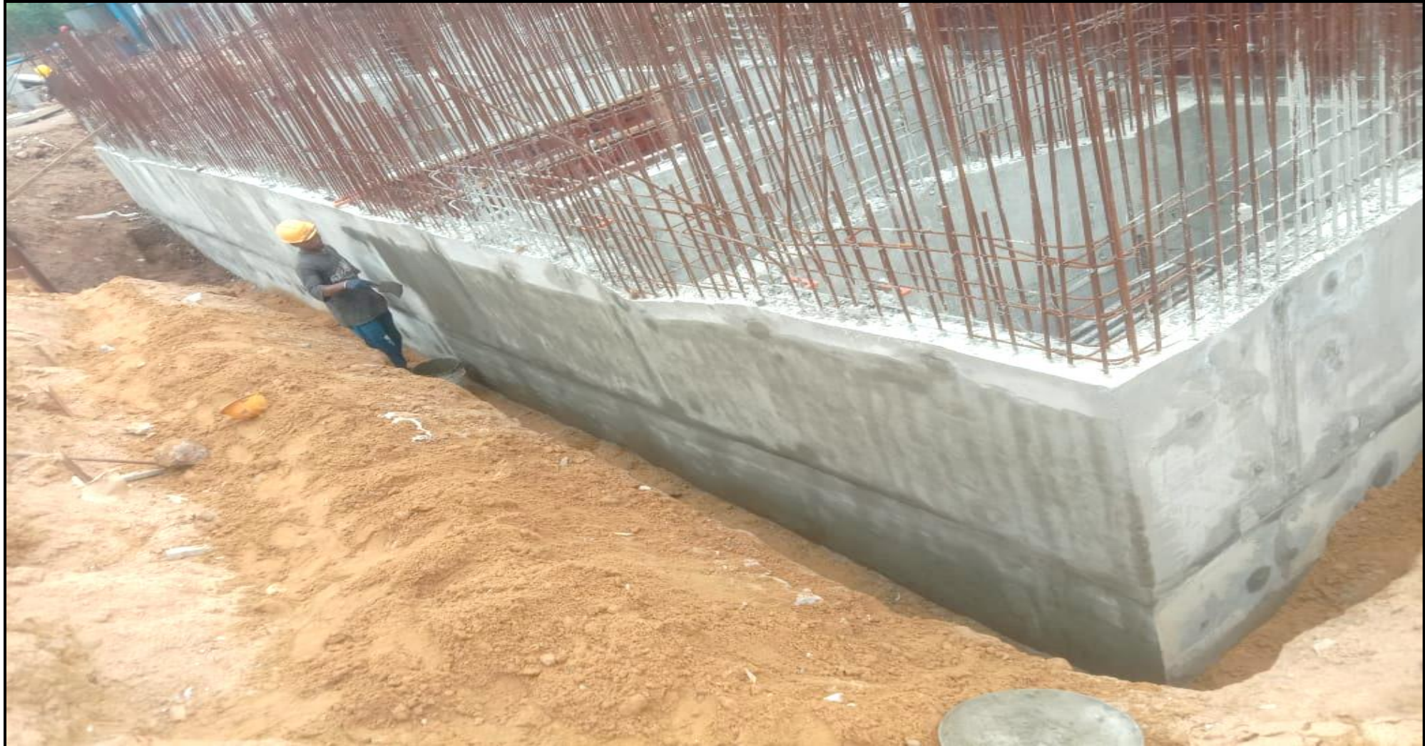
STP – External waterproofing work completed
