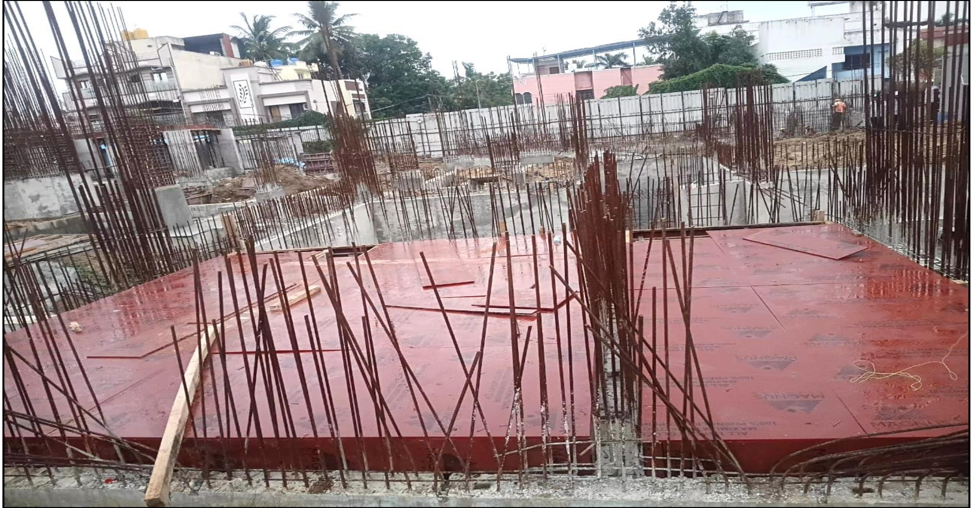
UG Sump – Cover slab shuttering work in progress
