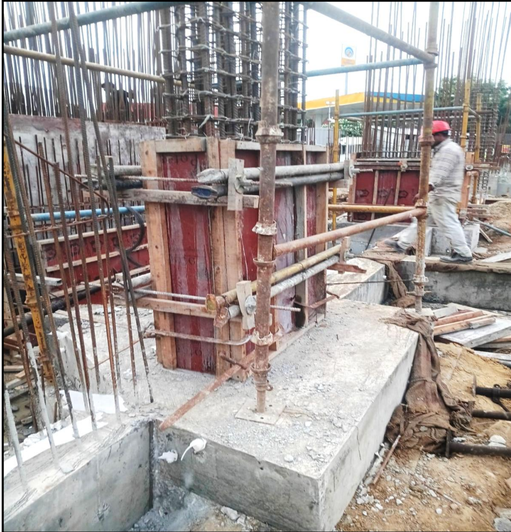
Main building – Stub column shuttering & concrete completed (47/47 Nos)
