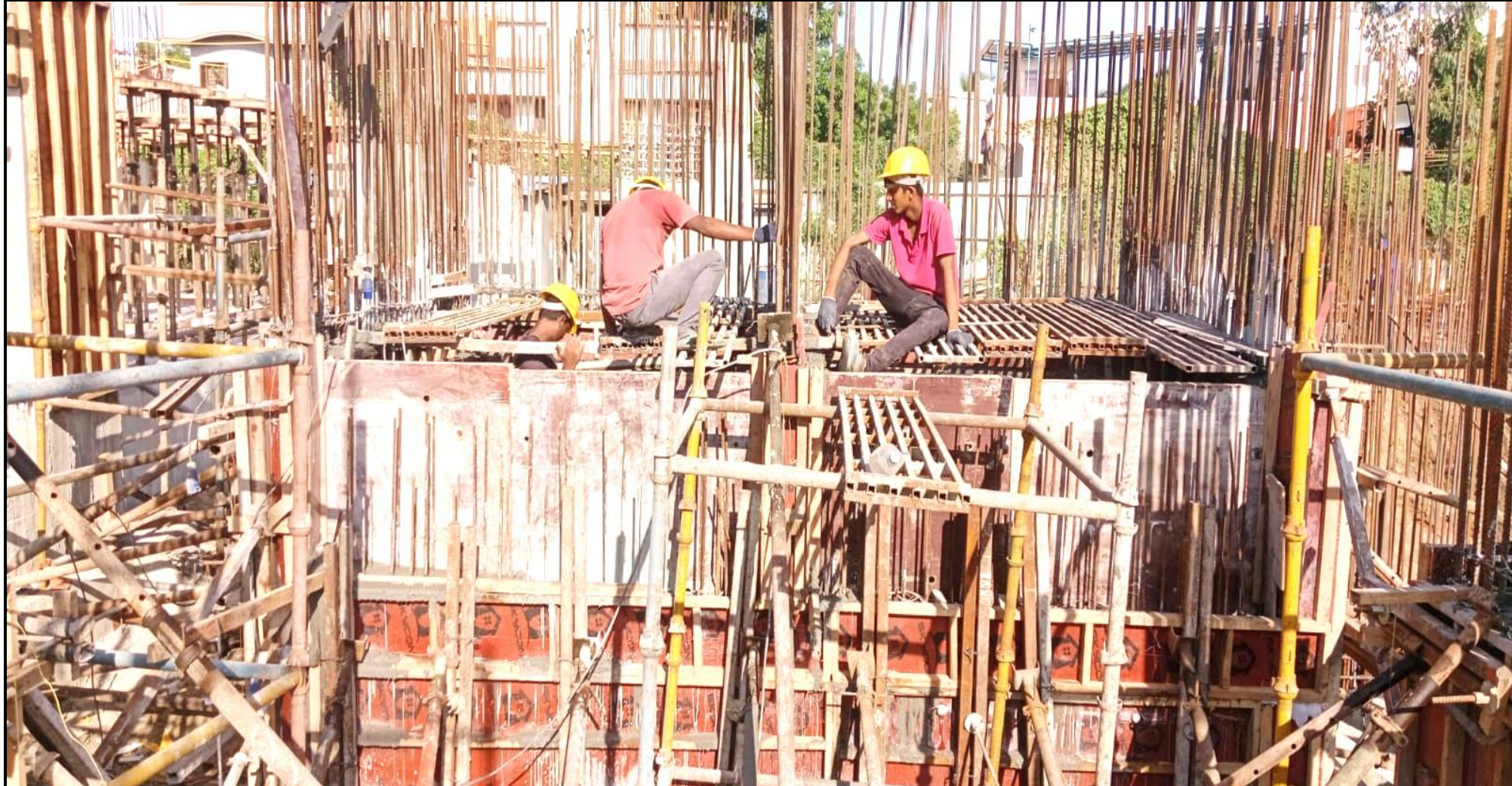
Main building – 1 st Lift core wall concrete completed
