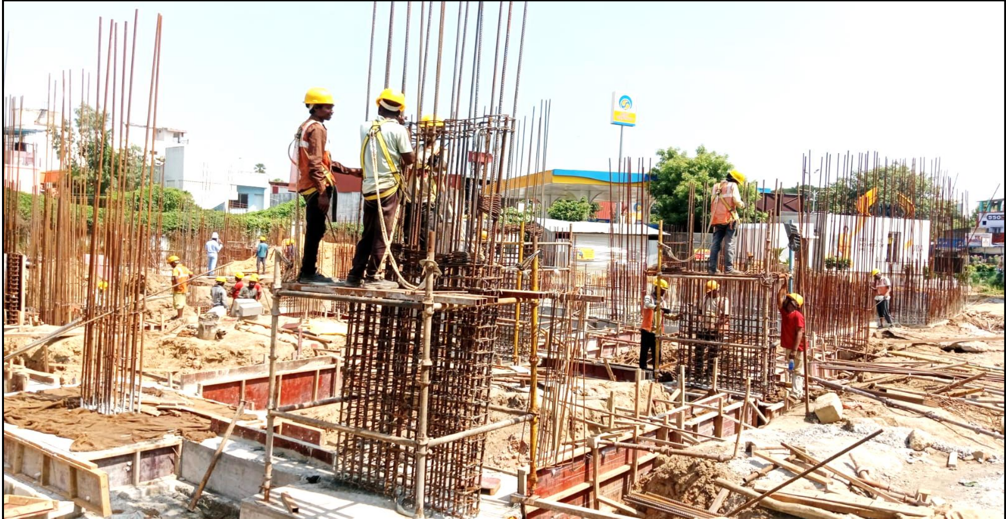
Main building – Stub column reinforcement completed (47/47 Nos)
