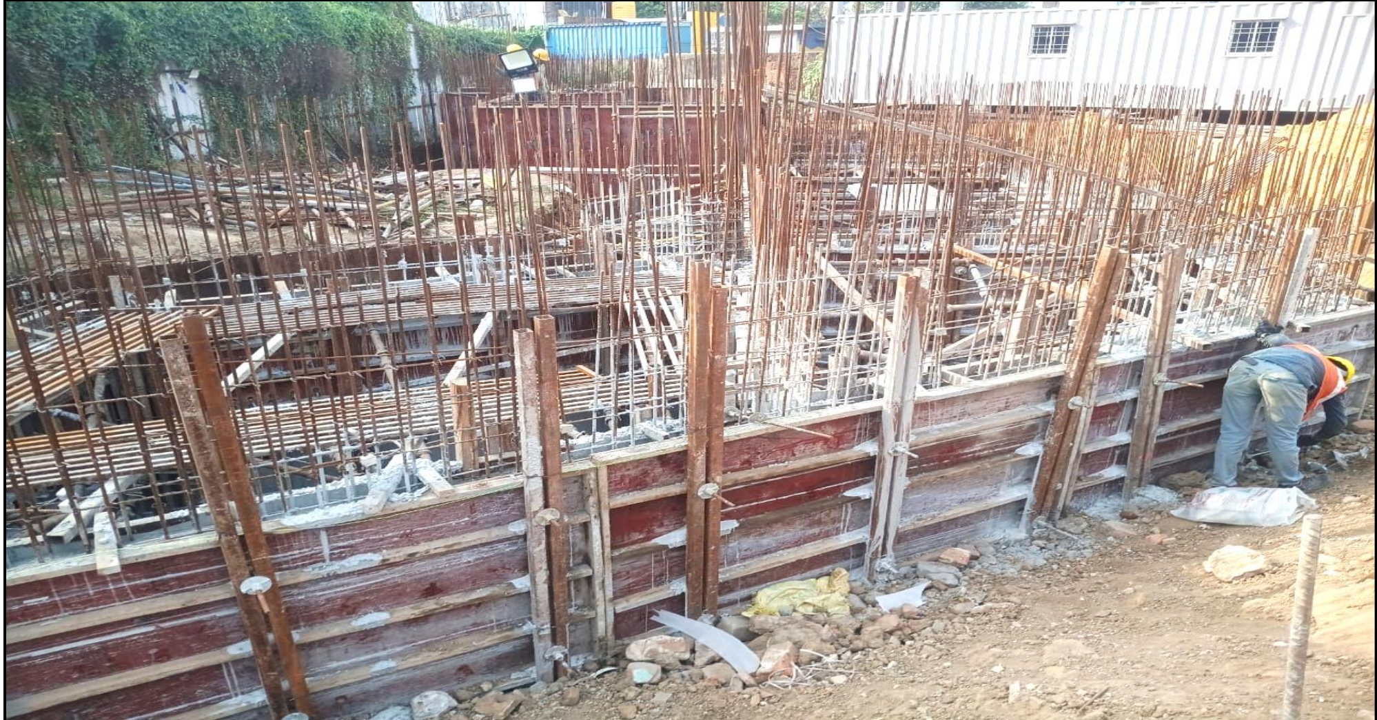
STP – 2 nd lift Wall concrete completed
