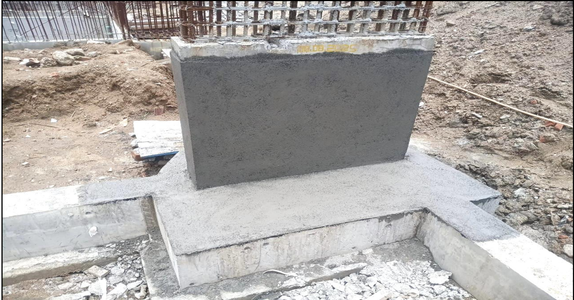
Main building – DPC on Pile cap, Plinth beam & Column completed (44/47 no's)
