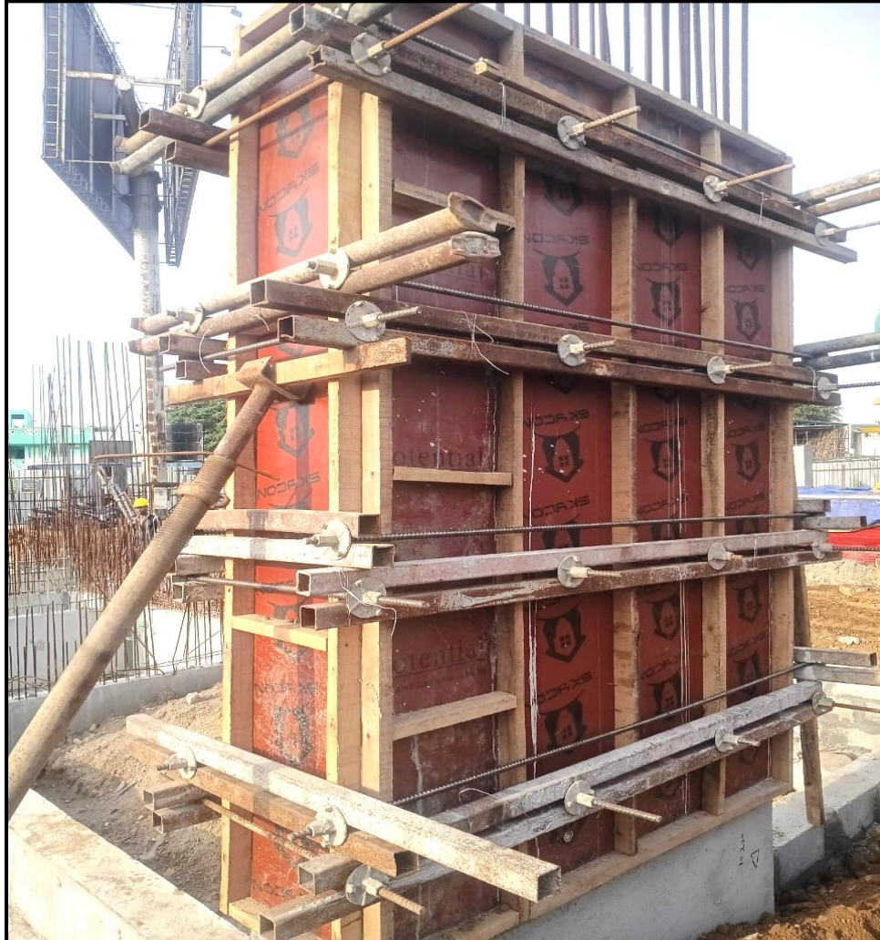
Main building – Pour 2 Stilt floor 2 nd lift column shuttering completed
