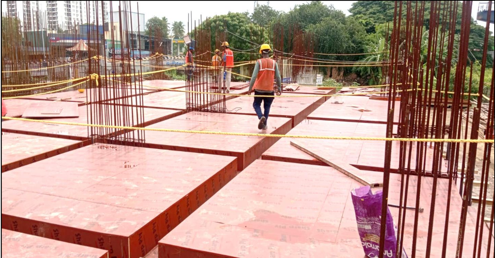
Main building – Pour 1 stilt floor roof slab shuttering work completed
