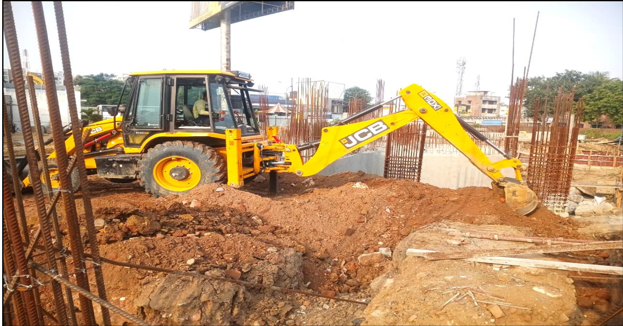
UG Sump – Back filling work in progress
