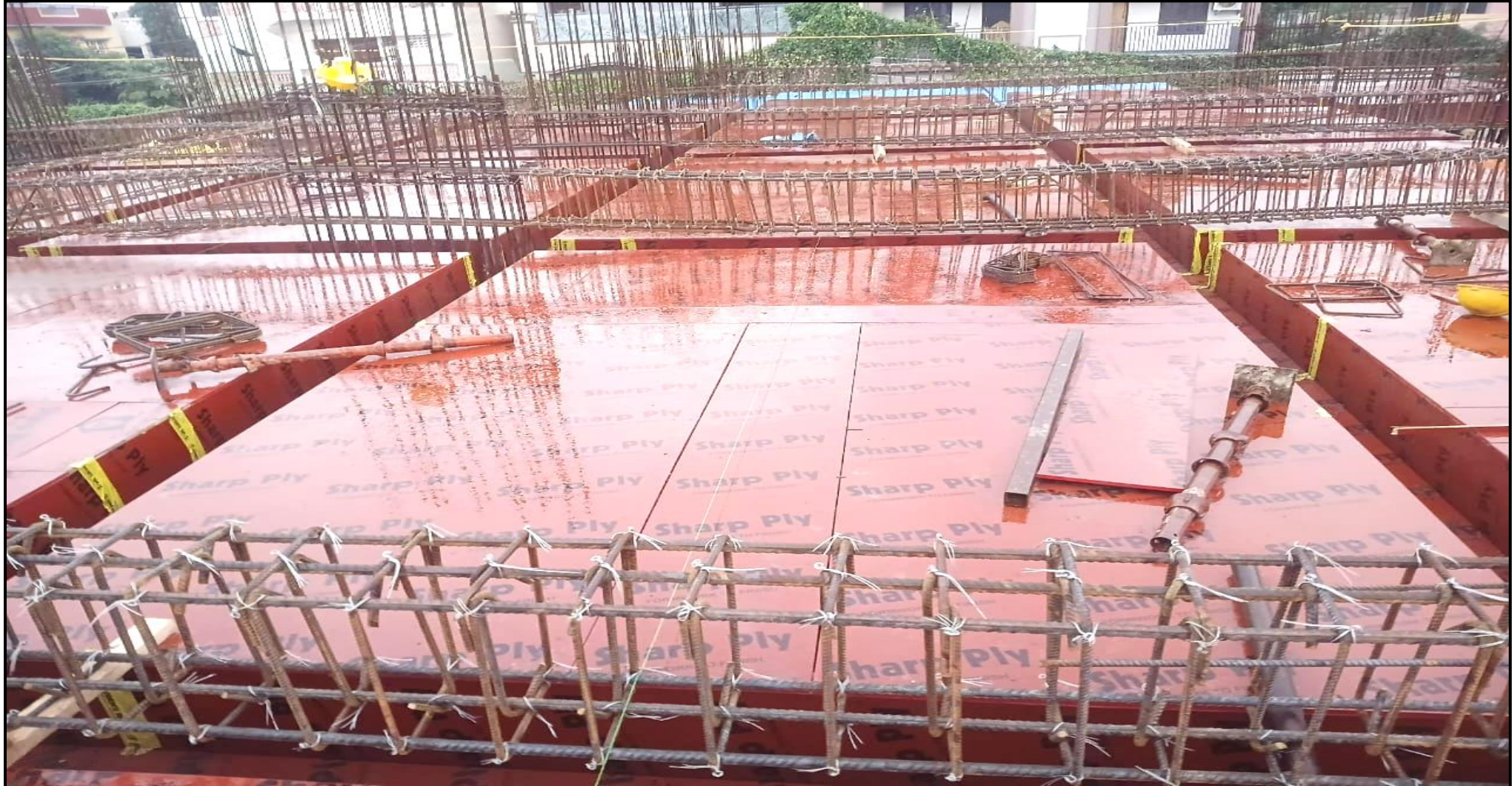
Main building – Pour 1 stilt floor roof beam reinforcement work completed
