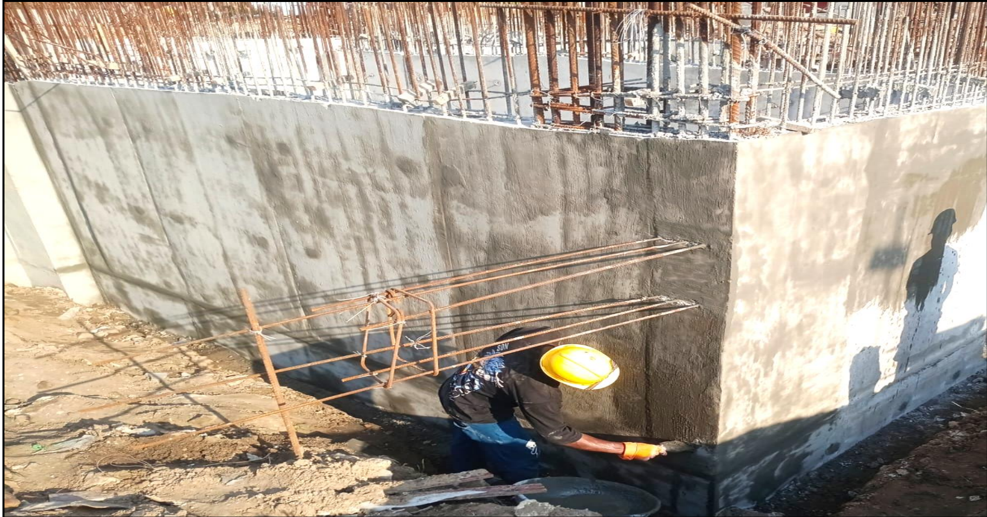
UG Sump – Waterproofing work completed
