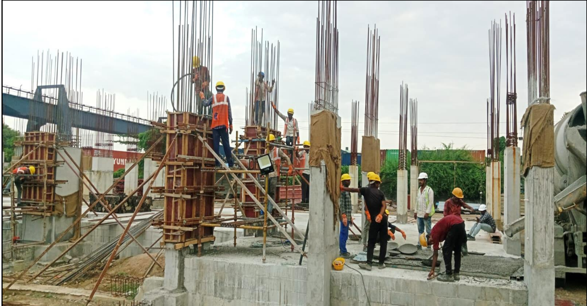
Main building – Stilt floor column 2 nd lift concrete completed (36/47nos)
