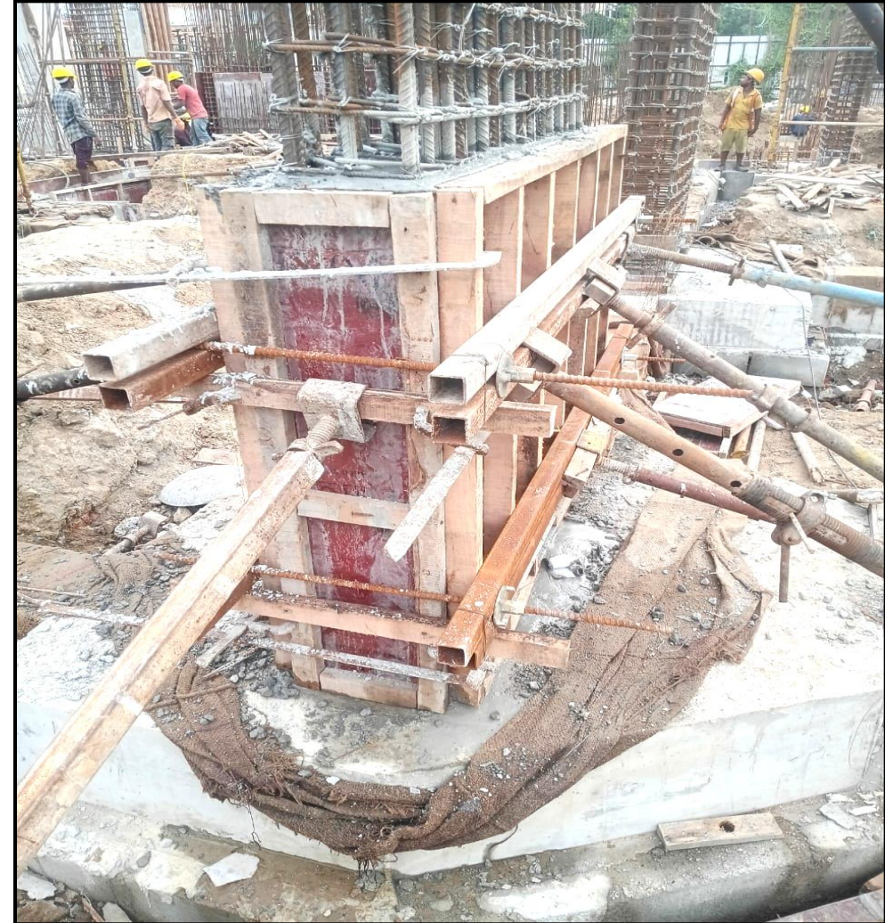
Main building – Stub column shuttering & concrete completed (47/47 Nos)
