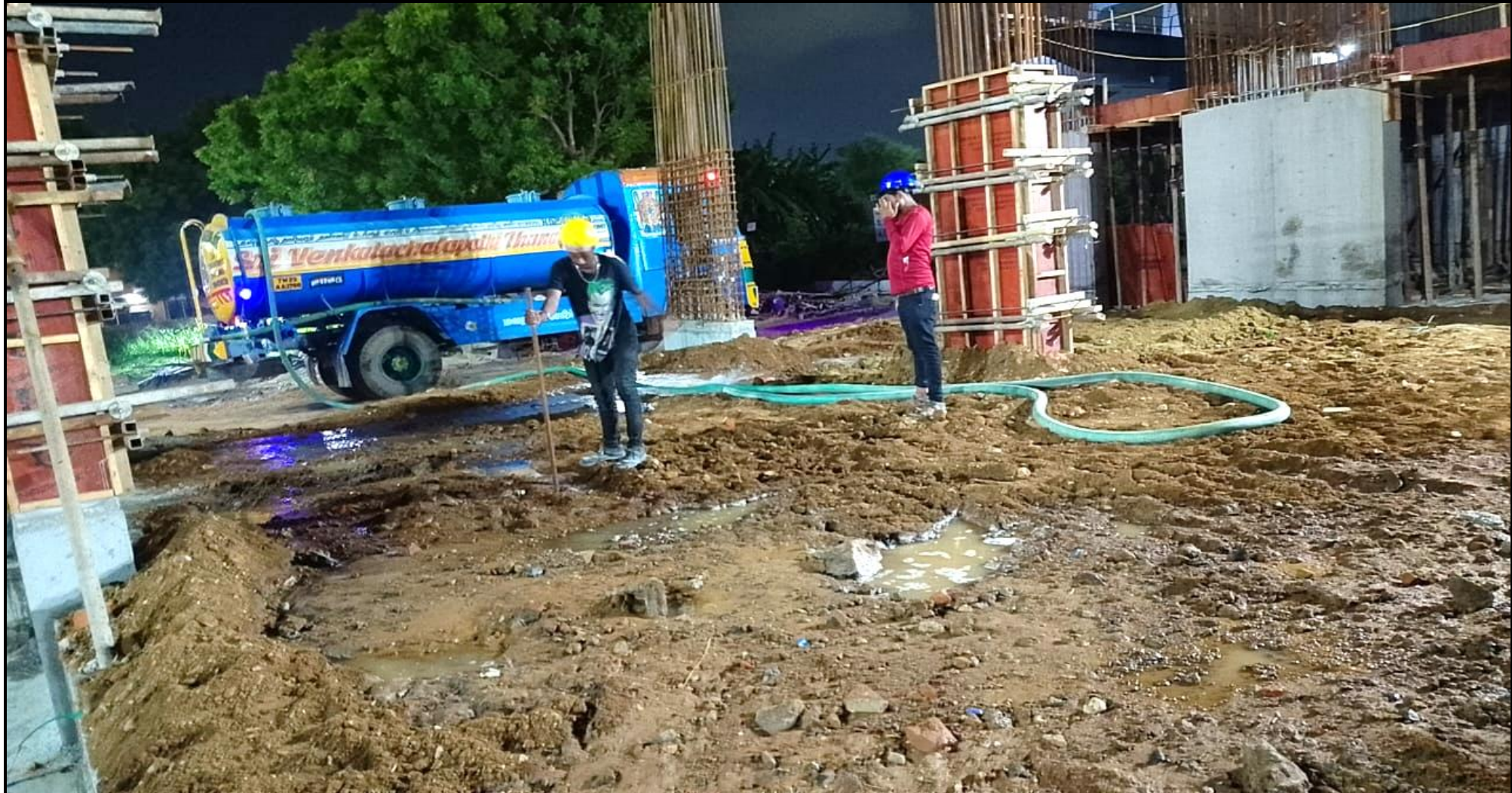
Main building – Pour 2 area Consolidation & soil levelling work in progress
