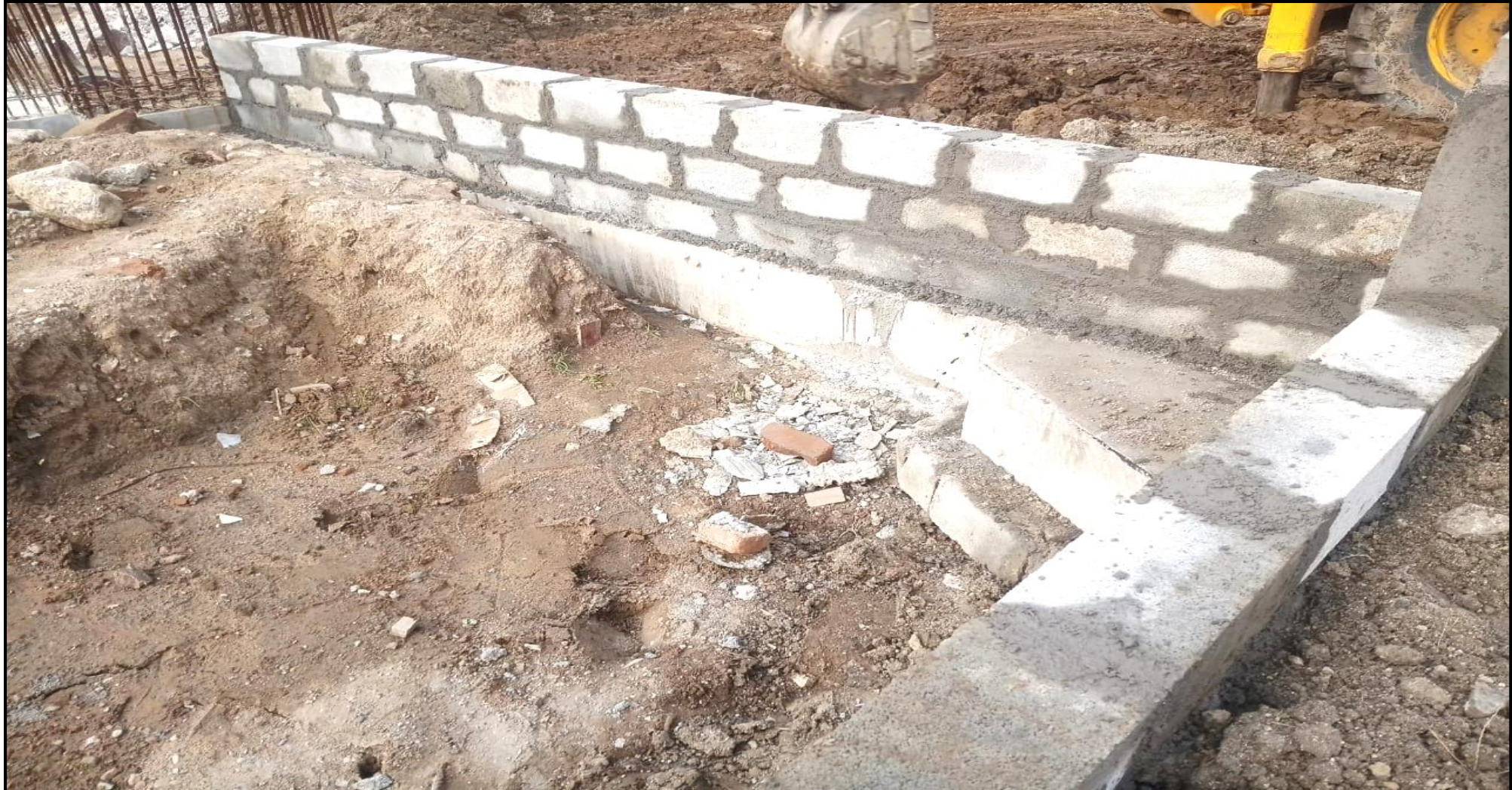
Main building – Pour 2 basement block work in progress
