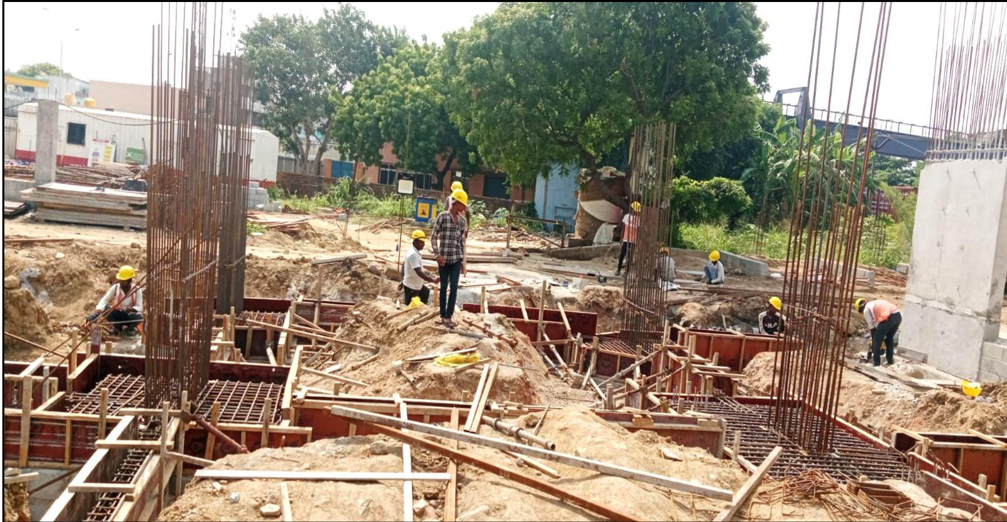
Main building – Pour 2 pile cap & plinth beam shuttering work completed
