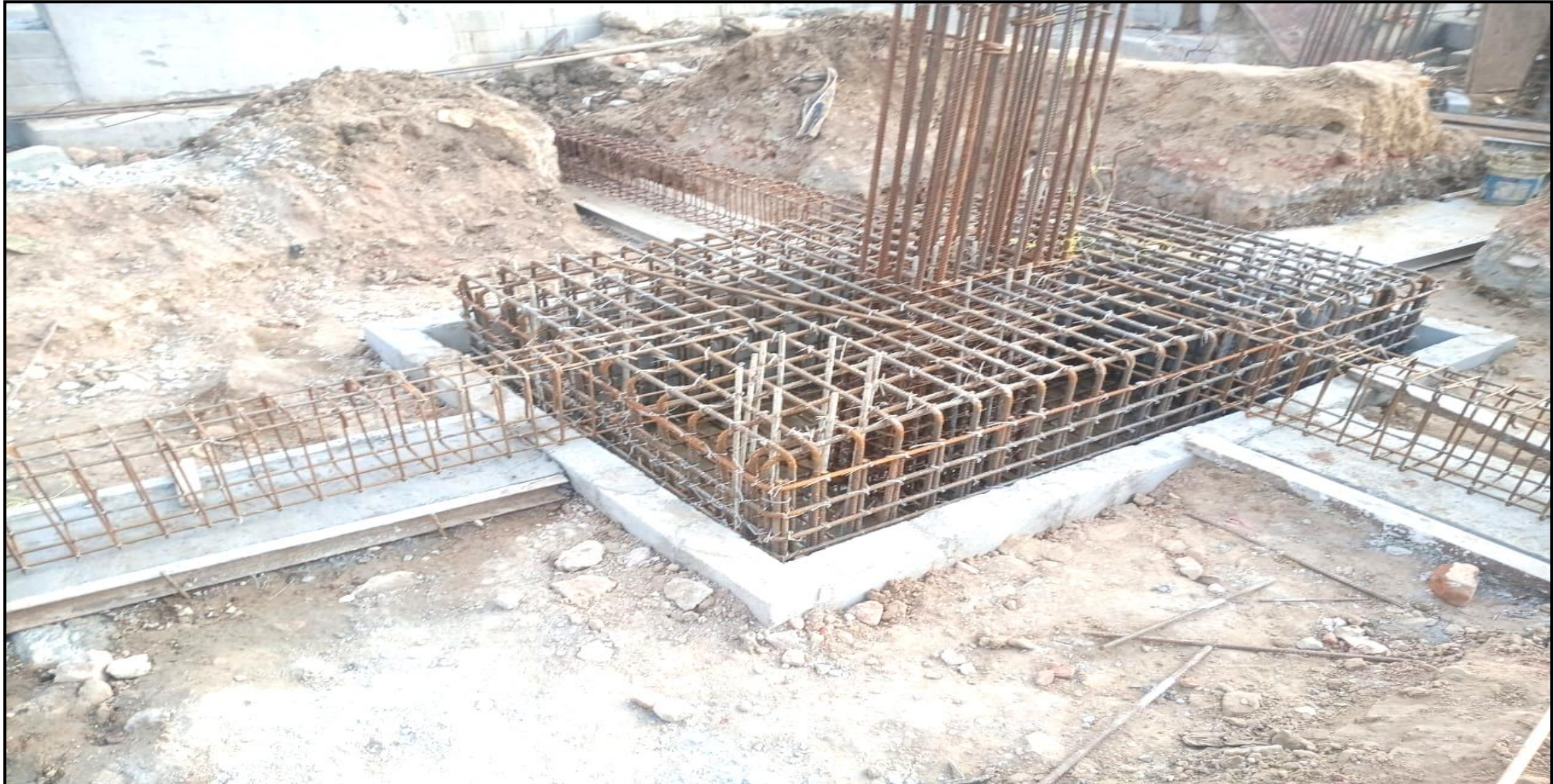
Main building – Pour 2 Pile cap & plinth beam reinforcement work completed
