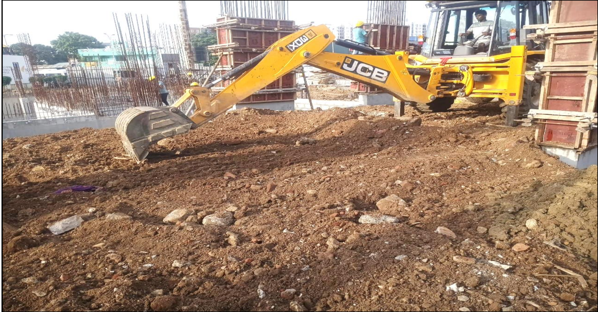
Main building – Pour 2 back filling work in progress
