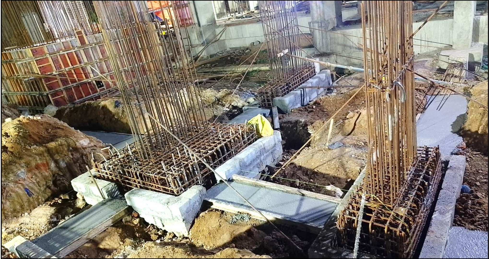
Main building – Pour 2 plinth beam PCC work completed
