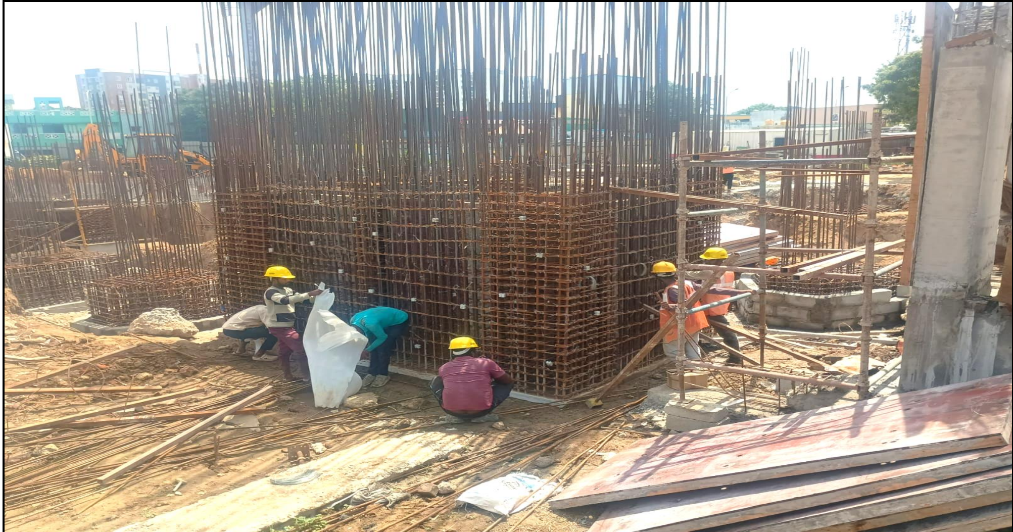
Main building – 1 st lift core wall reinforcement work completed
