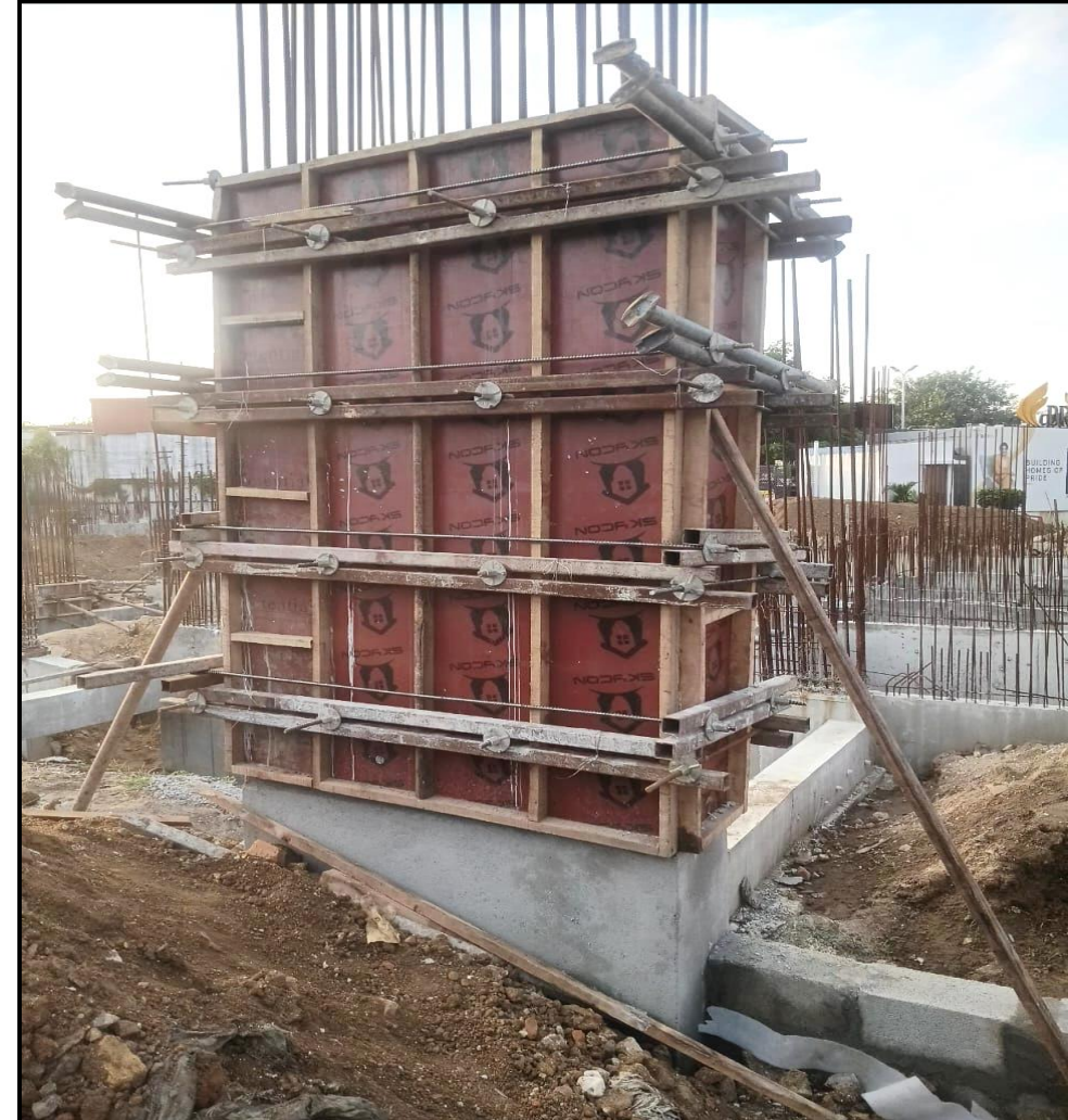
Main building – Pour 2 Stilt floor 2 nd lift column shuttering completed
