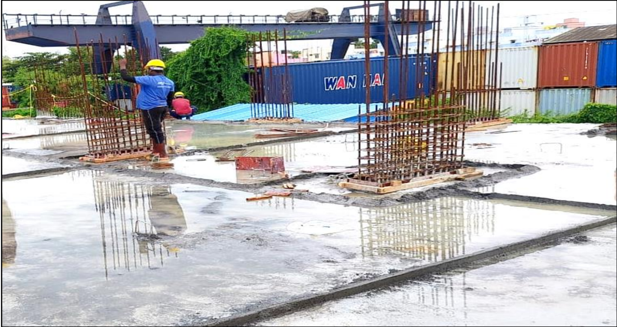
Main building – Pour 1 stilt floor roof slab curing bund making & curing work
