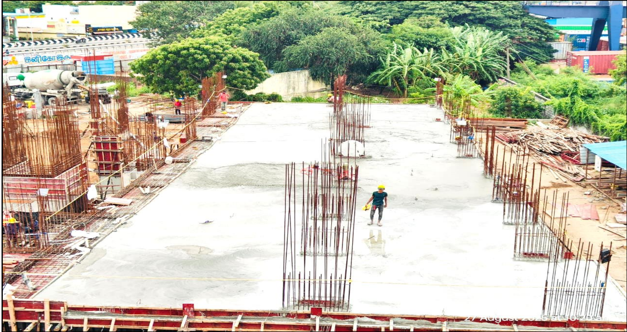
Main building – Pour 1 stilt floor roof slab concrete work completed
