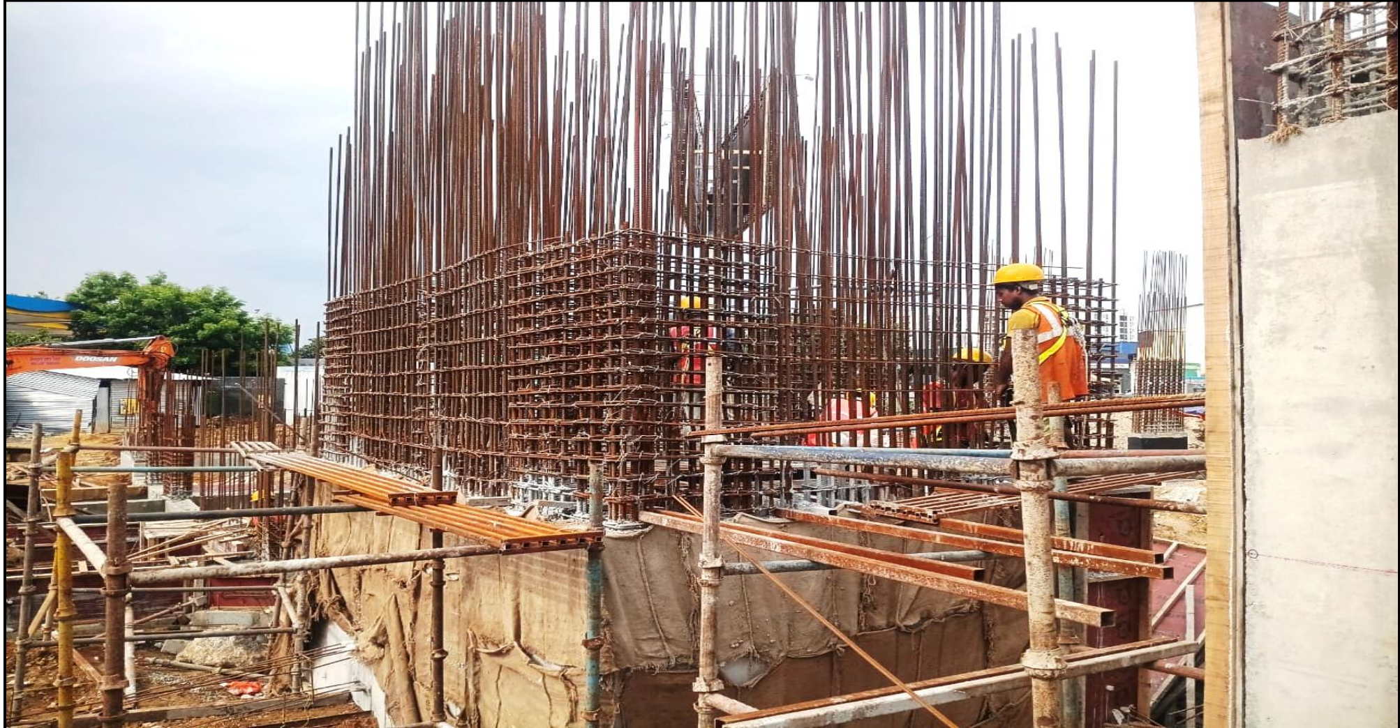
Main building – 2 nd lift core wall reinforcement work completed
