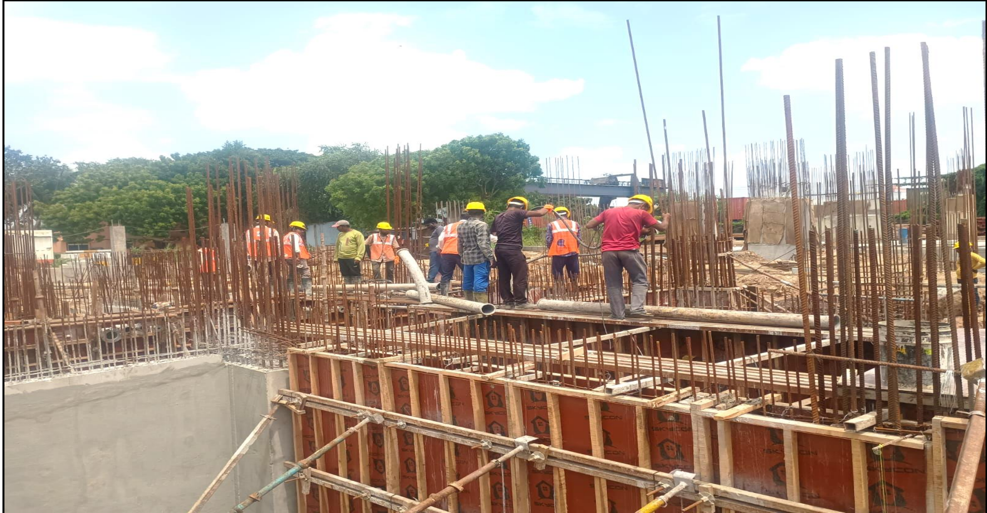
UG Sump – 2 nd lift Wall concrete work completed
