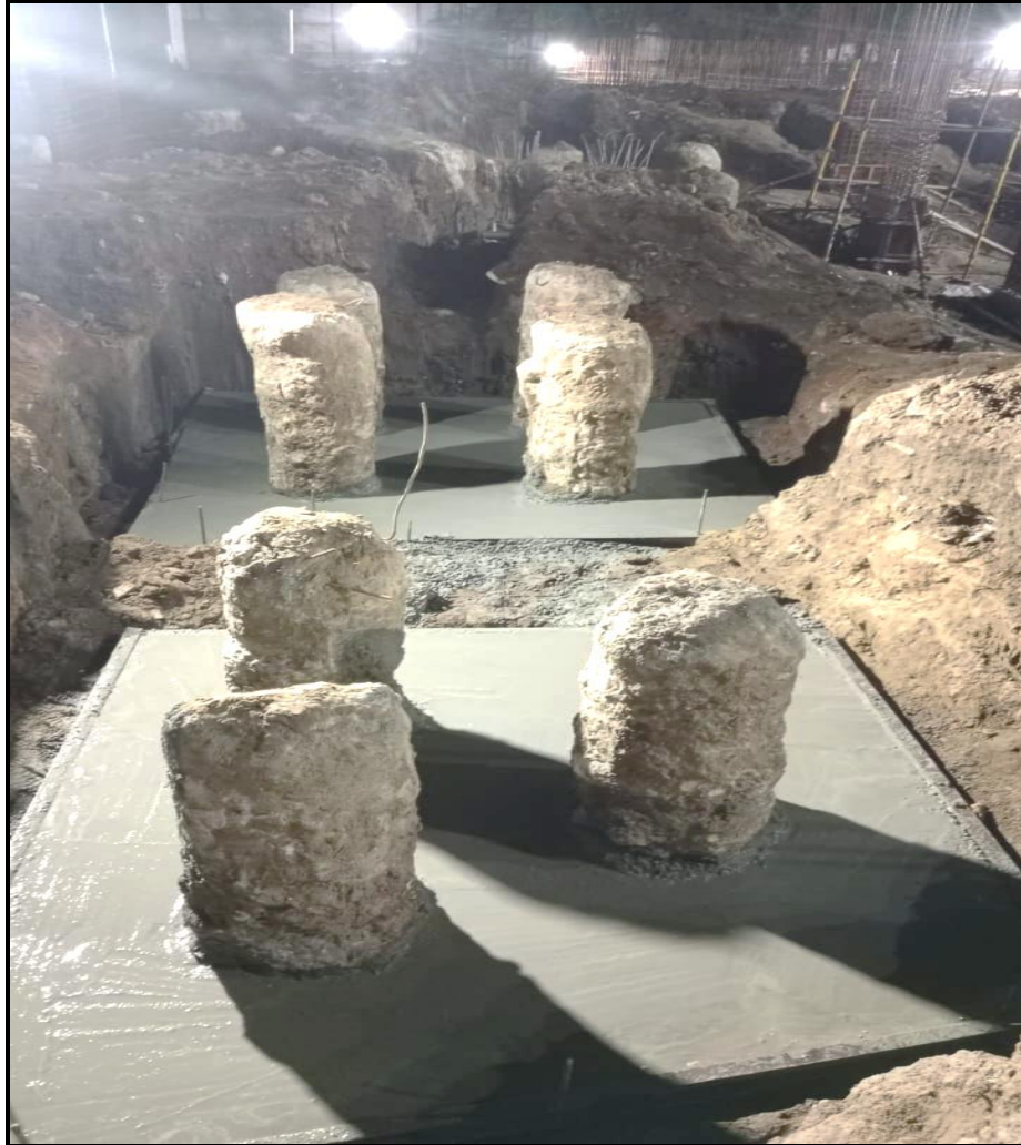
Main building – Pile cap pcc 15 no's completed (65/65 no's)
