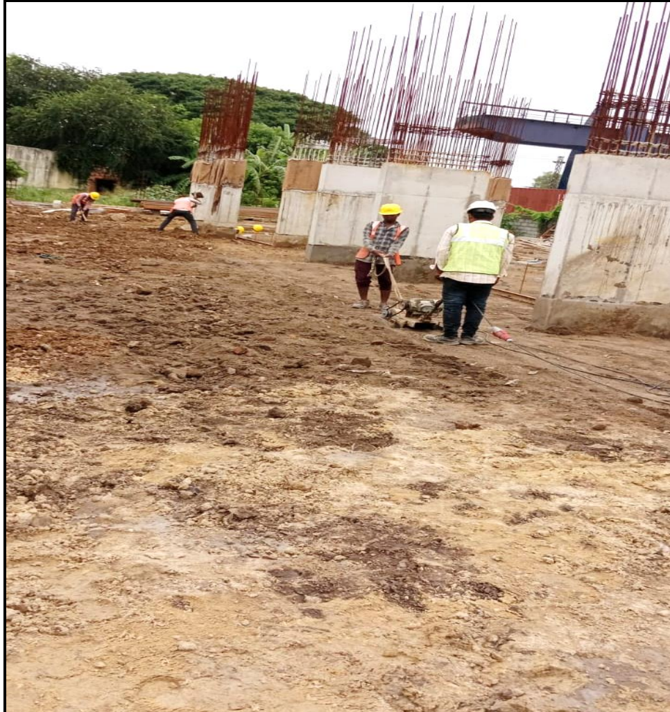
Main building – Surface dressing & compaction for grade slab PCC
