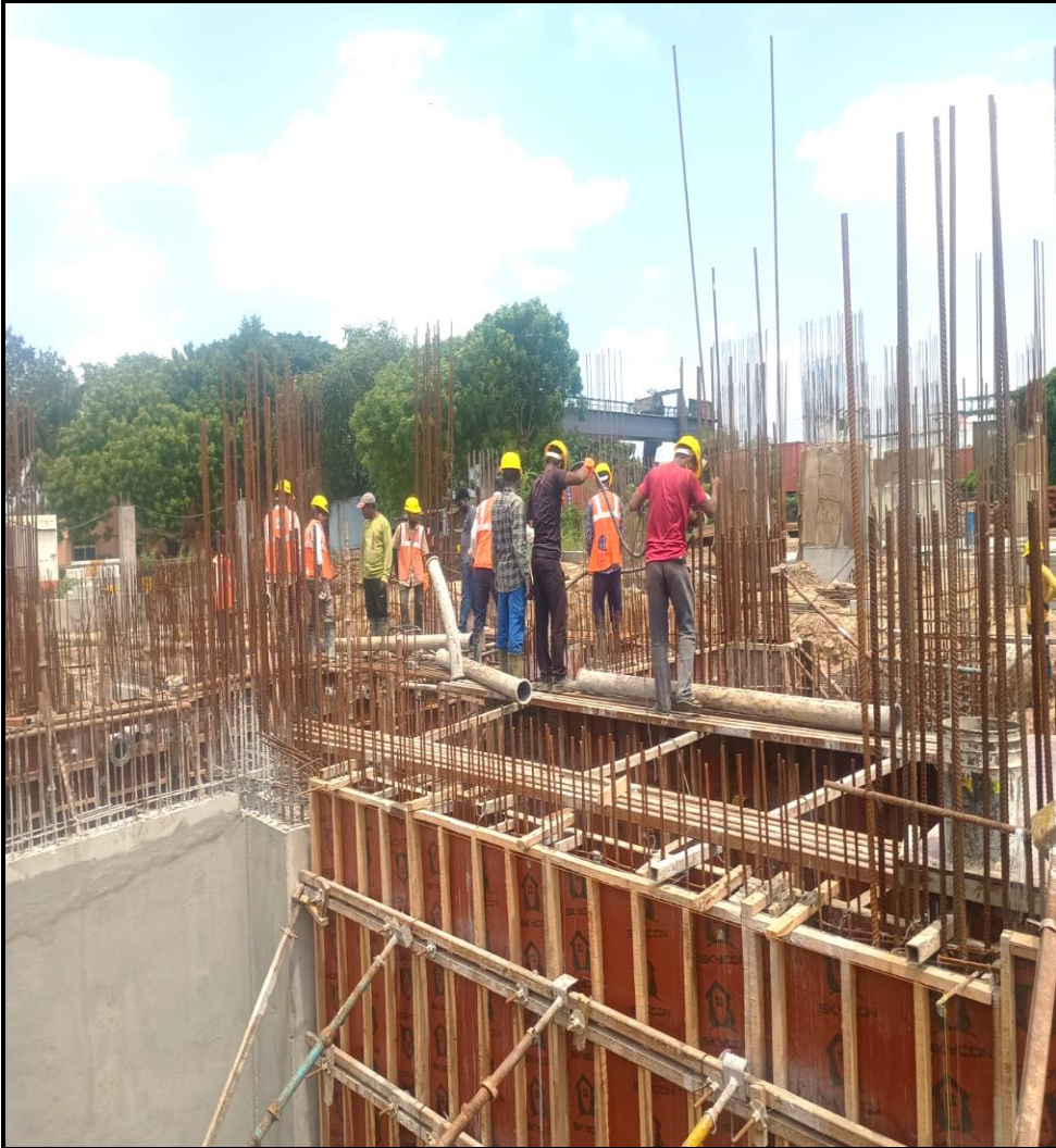
UG Sump – 2 nd lift wall concrete completed
