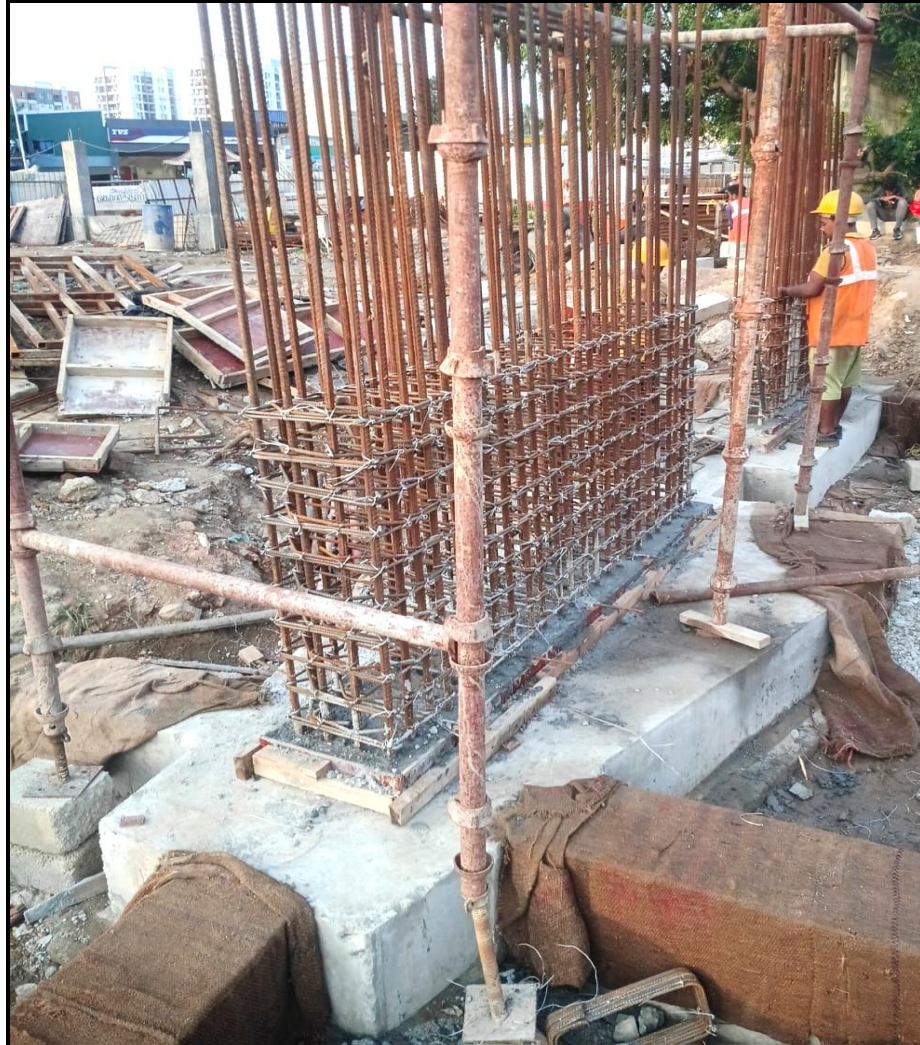
Main building – Column starter concrete and 1 st lift reinforcement work completed
