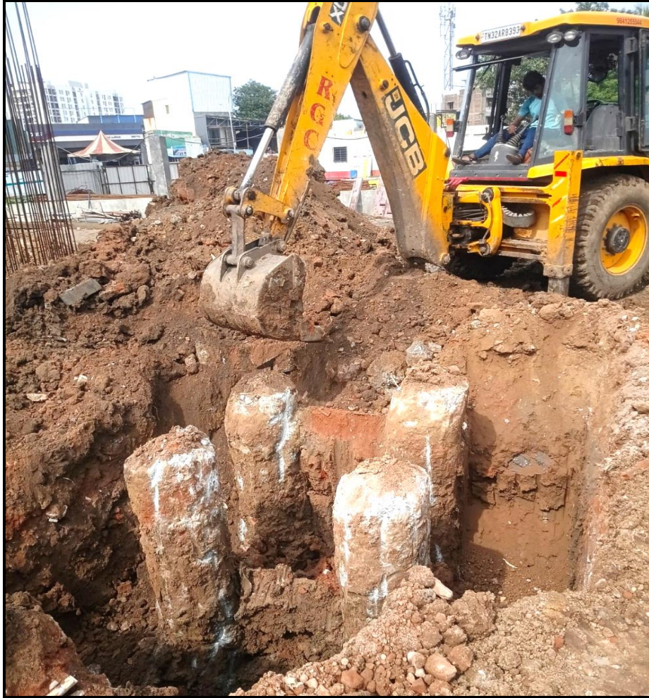
Main building – Pile cap excavation work 15 no's completed (65/65 no's)
