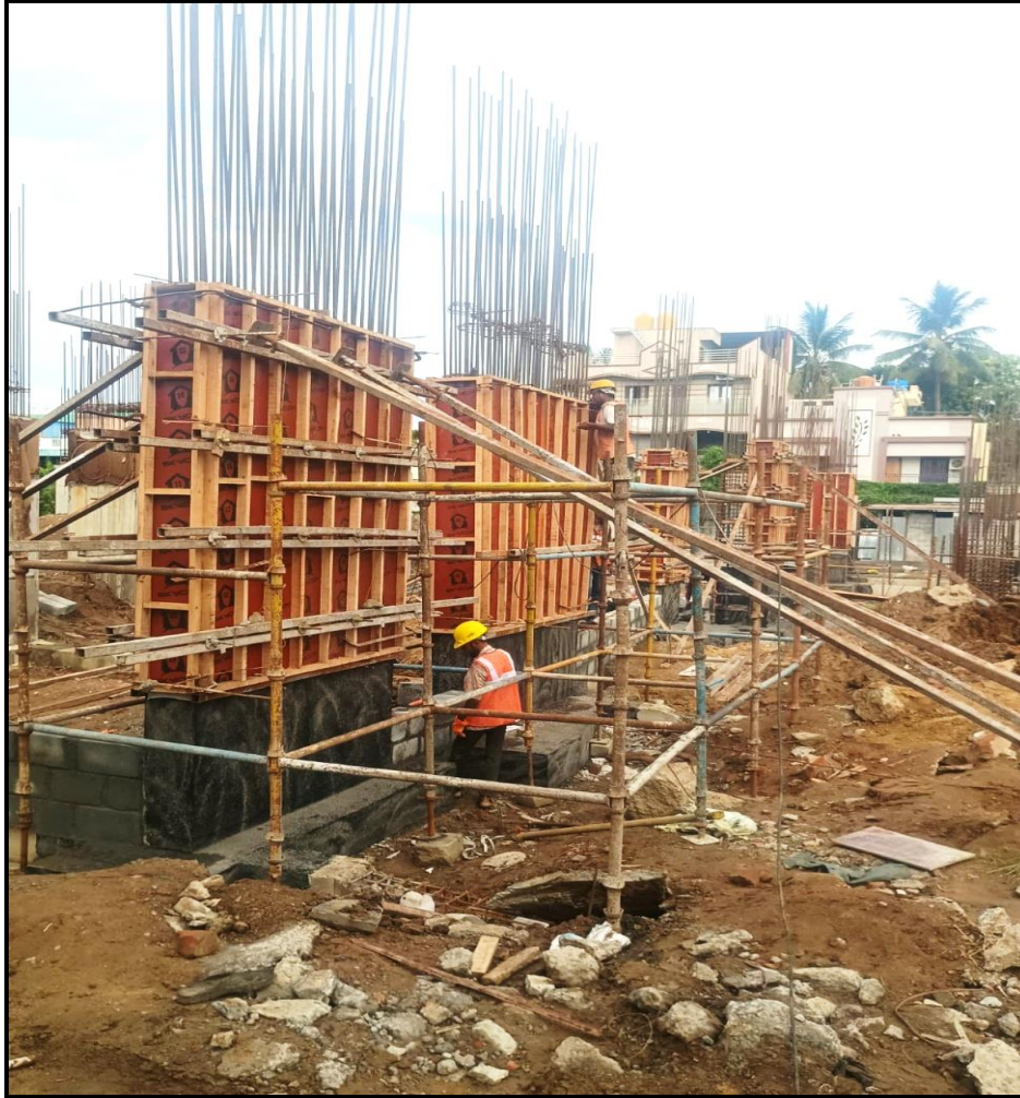
Main building – Stilt floor column 1 st lift shuttering 7 no's completed (49/65 no's)
