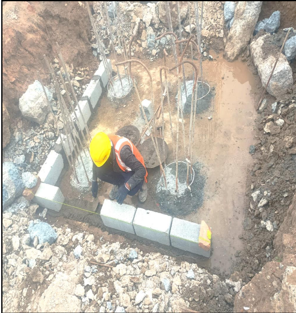
Main building – Pile cap block work in progress
