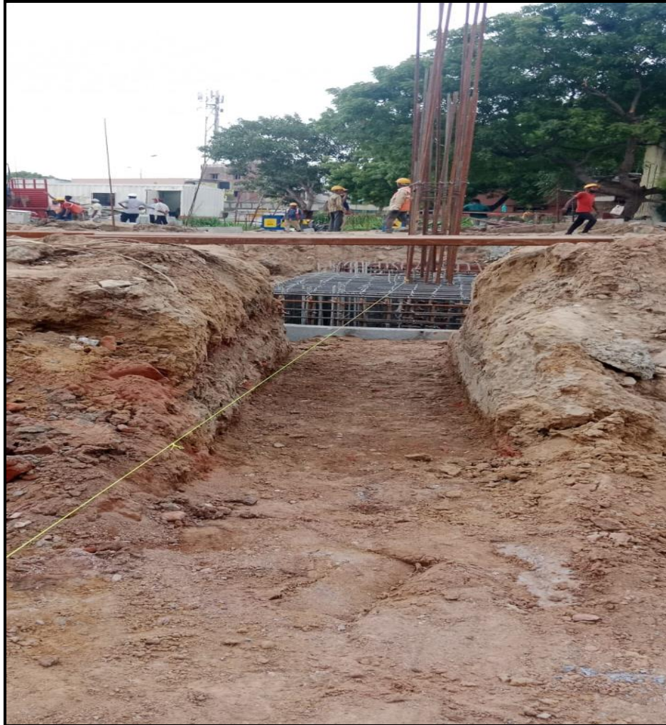
Main building – Plinth beam base dressing for pcc (197/285 m)
