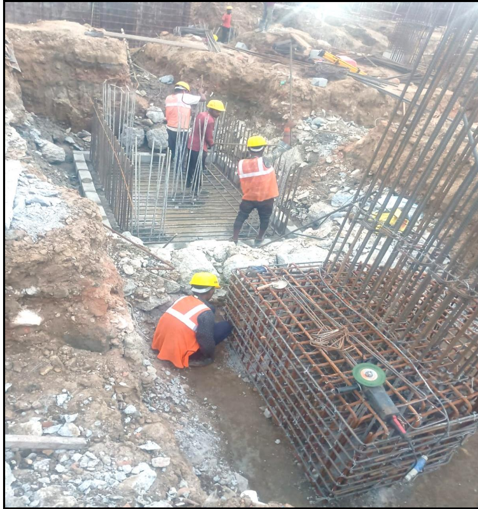
Main building – Pile cap reinforcement work 10 no's completed (40/47 nos)
