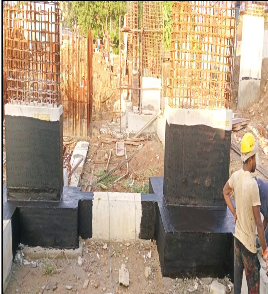
Main building – DPC coating & protective plastering on column completed (30/47 no's)
