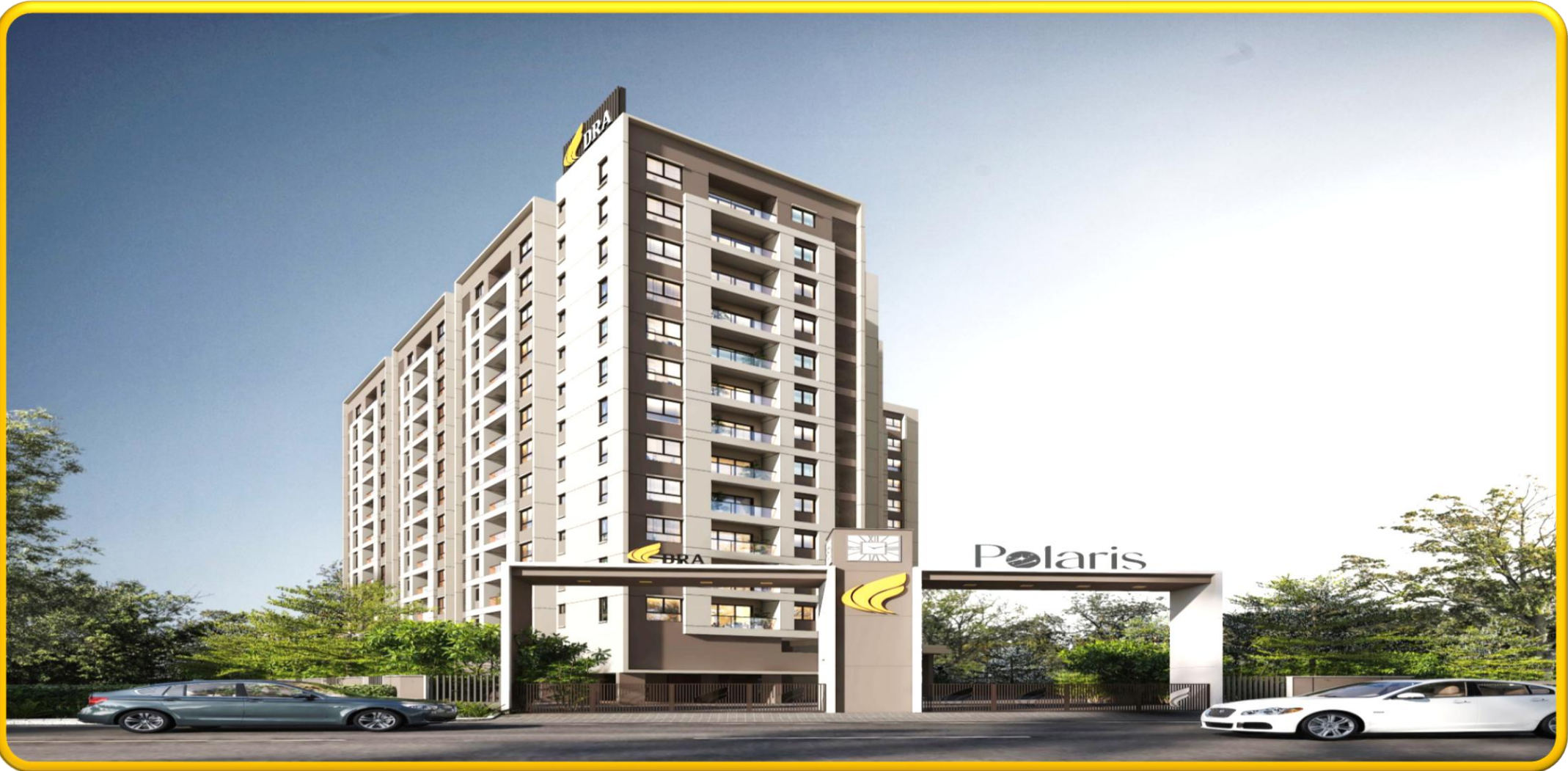
DRA POLARIS Construction updates photos – October 2025
